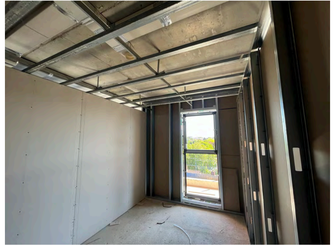
Metal ceiling grid installation ongoing
