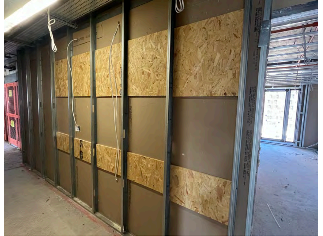
1 st side boarding of walls and pattress installation ongoing
