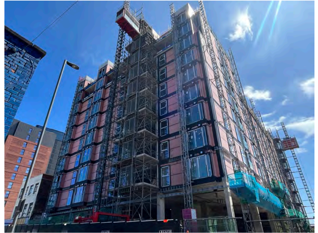
Block D Section B – Weatherboarding
