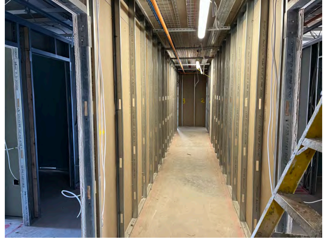
1 st side boarding ongoing
