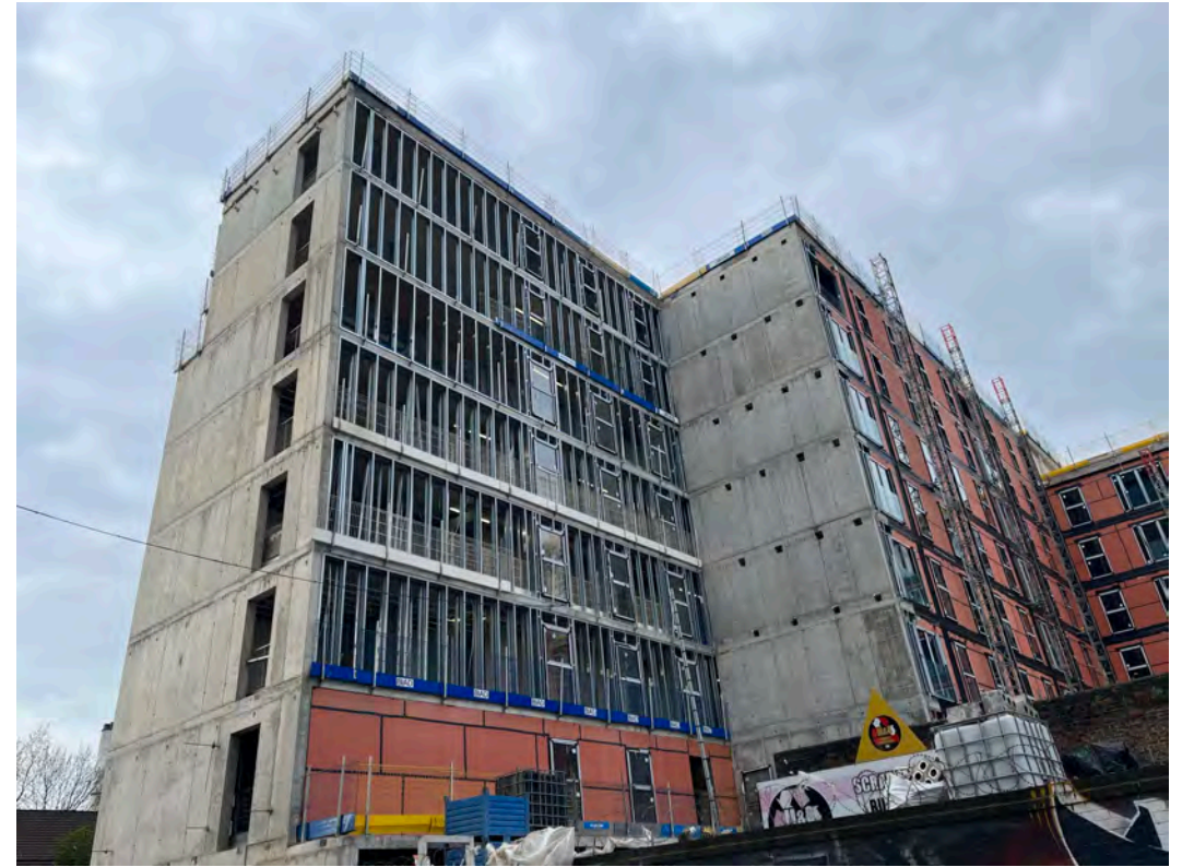
Block D Section B – SFS Installation
