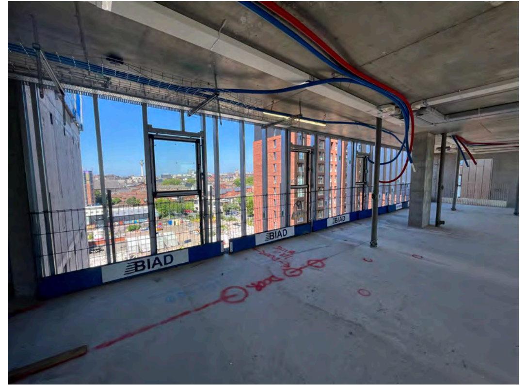
Apartment setting out ongoing
