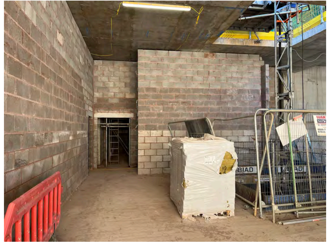
Ground Floor Internal blockwork ongoing
