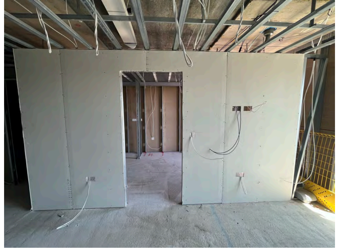
1 st fix electrical installation and 1 st side boarding ongoing
