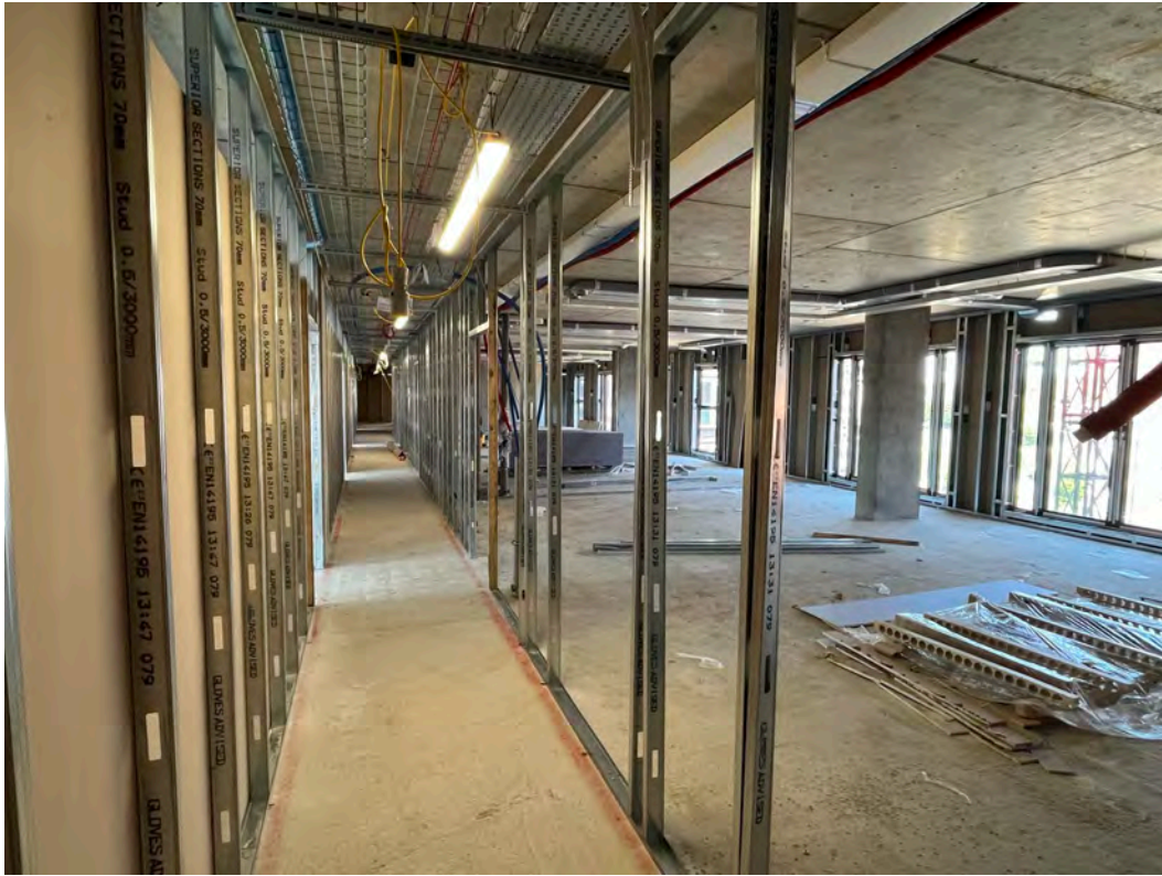
Partition wall installation ongoing
