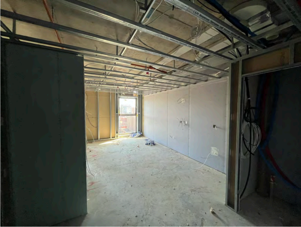
1 st side boarding of walls and metal ceiling grid installation ongoing
