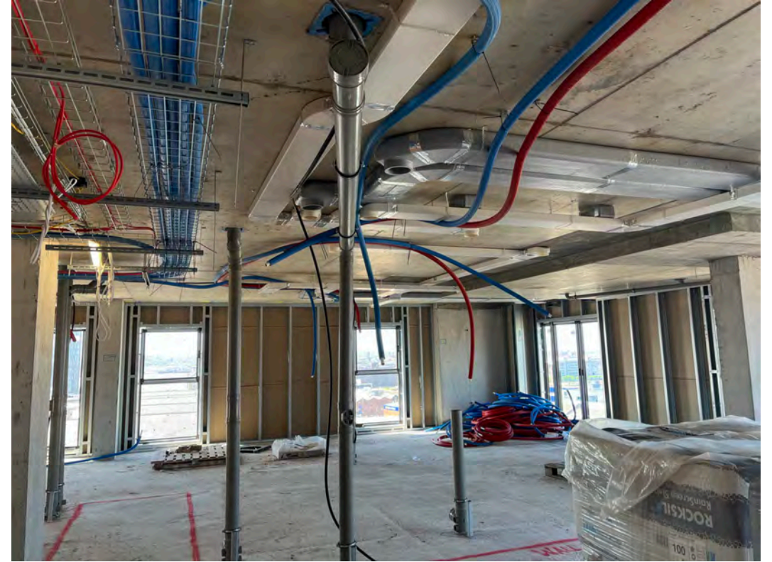
Apartment 1 st fix mechanical installation ongoing
