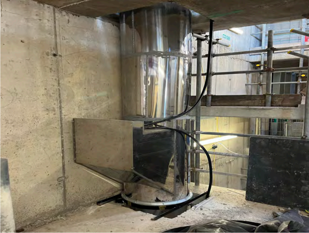
Bin chute installation
