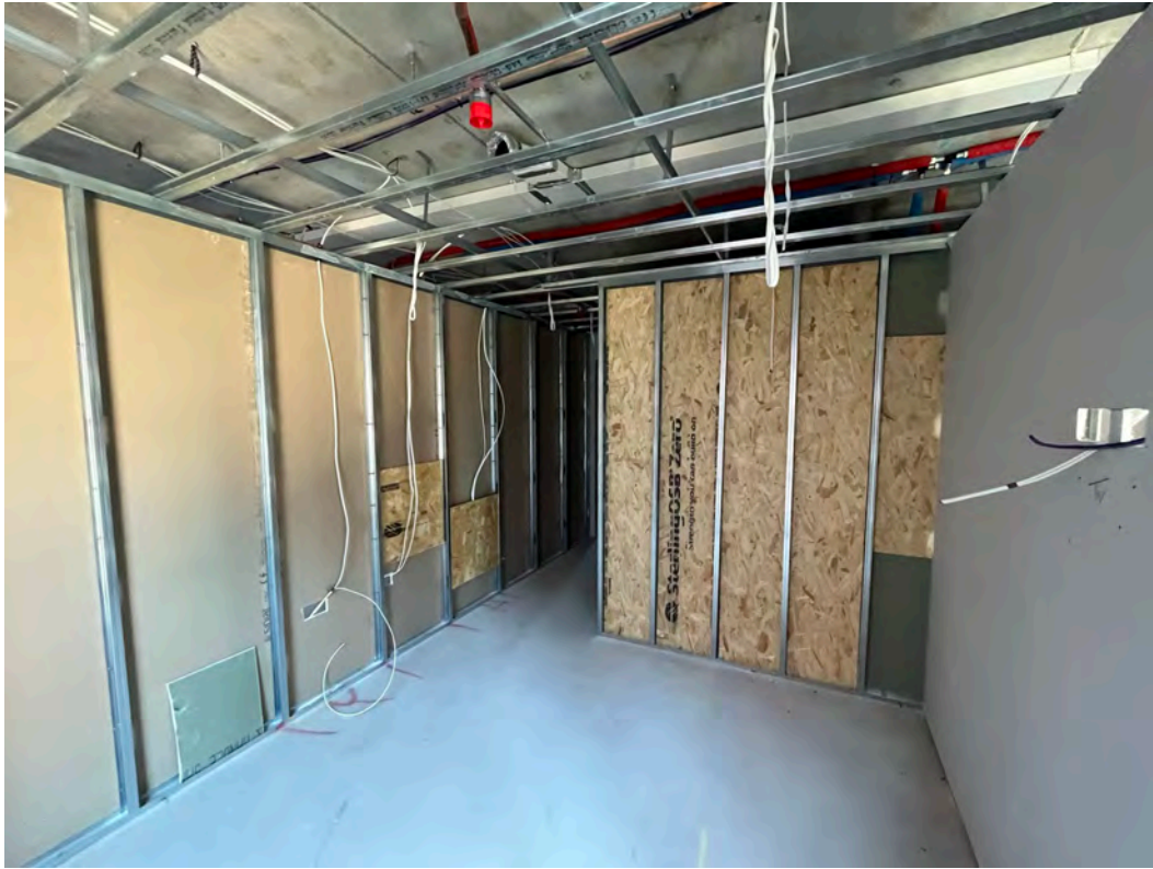
Pattress installation ongoing
