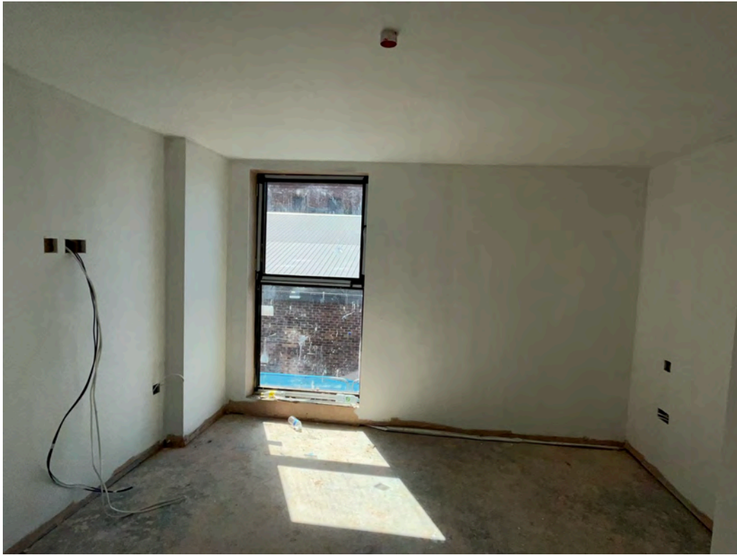
Mistcoat application ongoing
