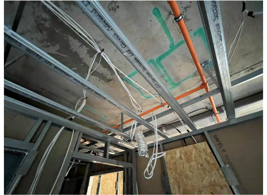
1 st fix electrical installation ongoing
