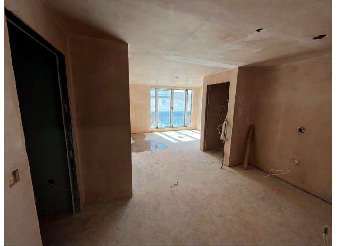
Plaster skim walls and ceiling application ongoing
