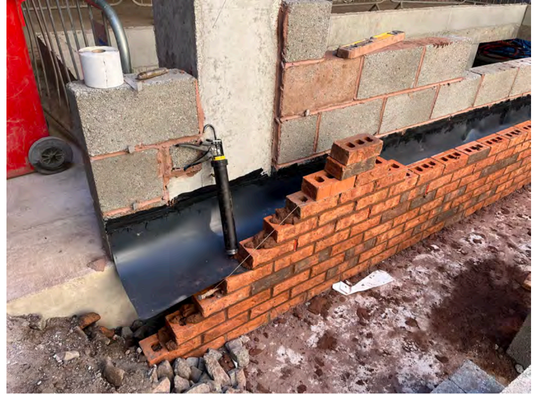
Ground floor cavity tray installed
