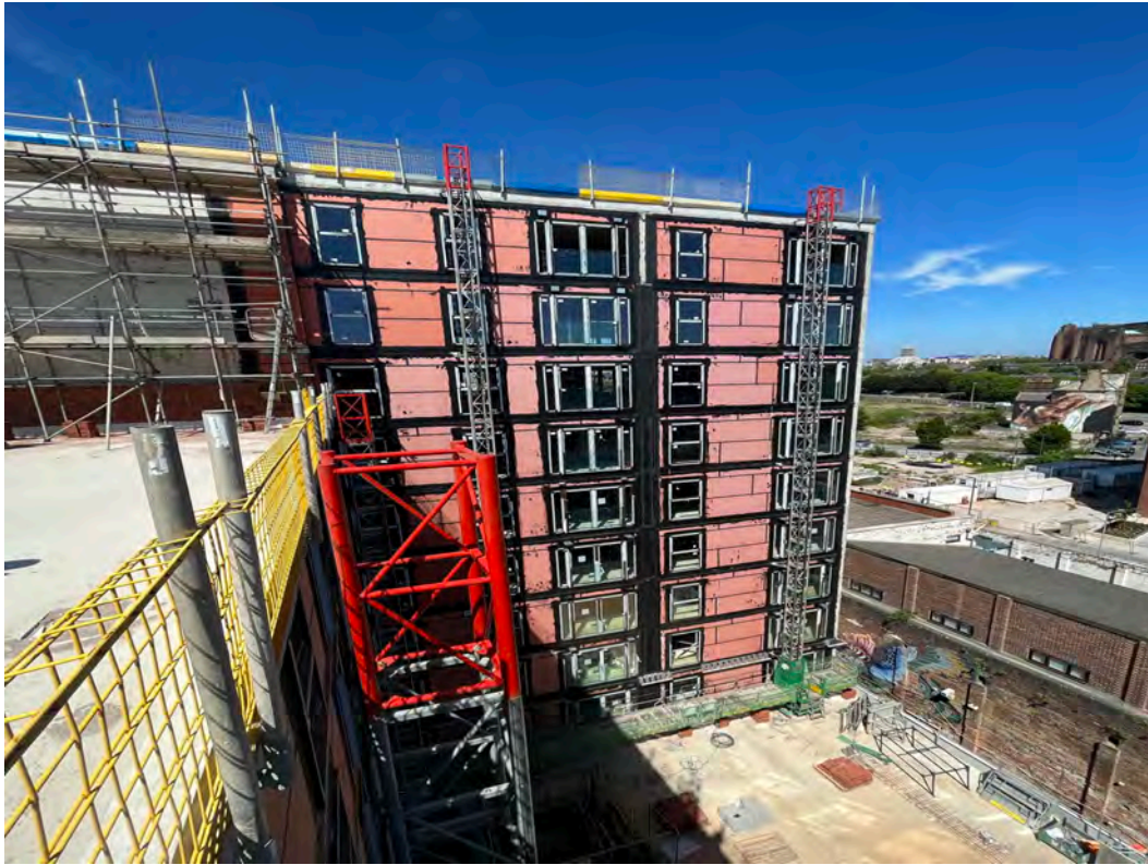
Block D Section A – SFS & Weatherboarding Installation
