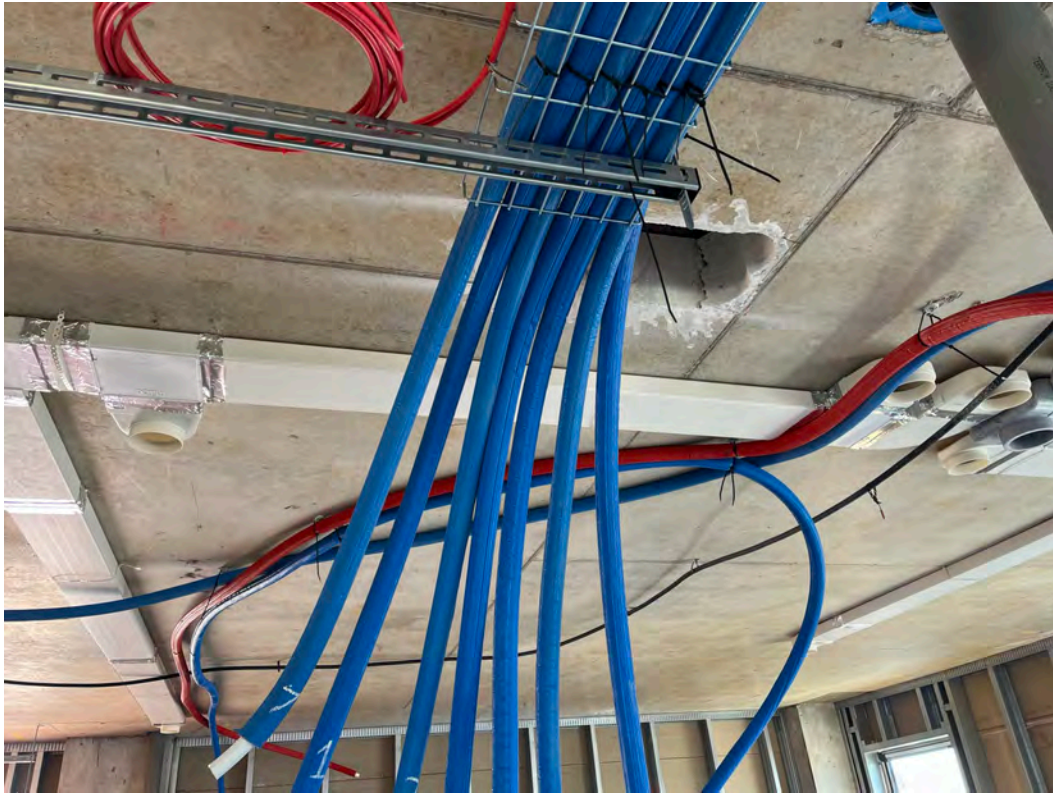
1 st fix mechanical hot and cold water feeds installation ongoing
