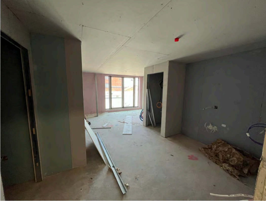
2 nd side boarding of walls and ceiling ongoing
