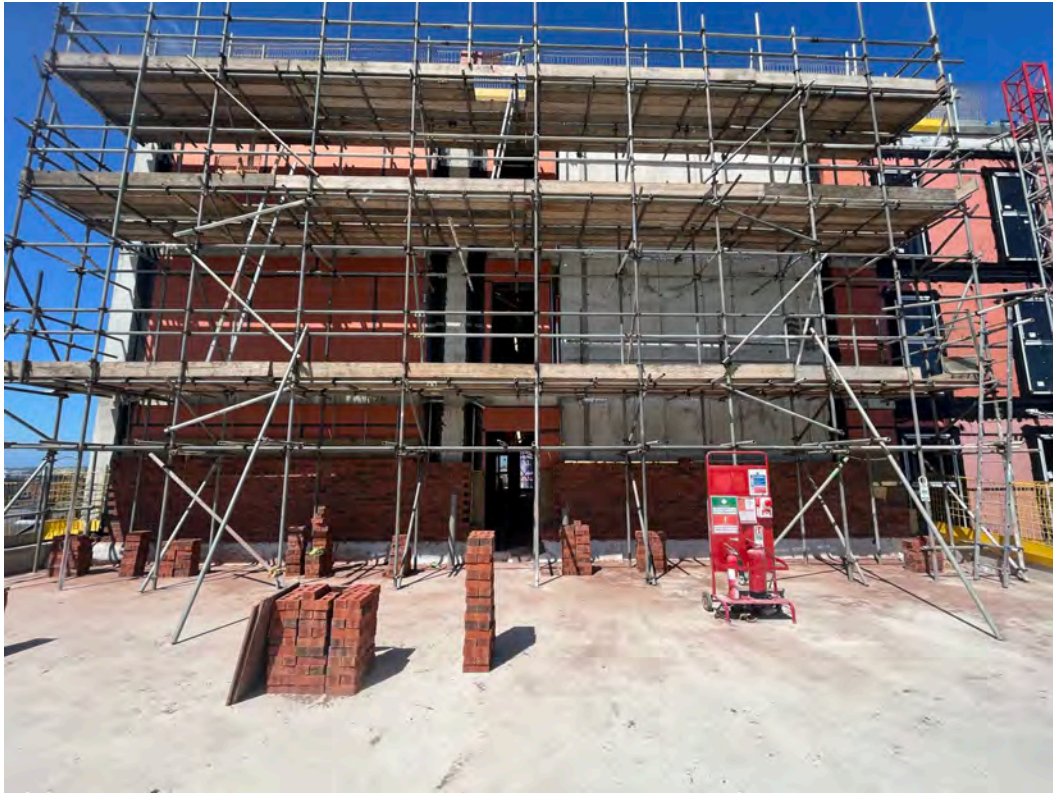
Block D – External brickwork ongoing
