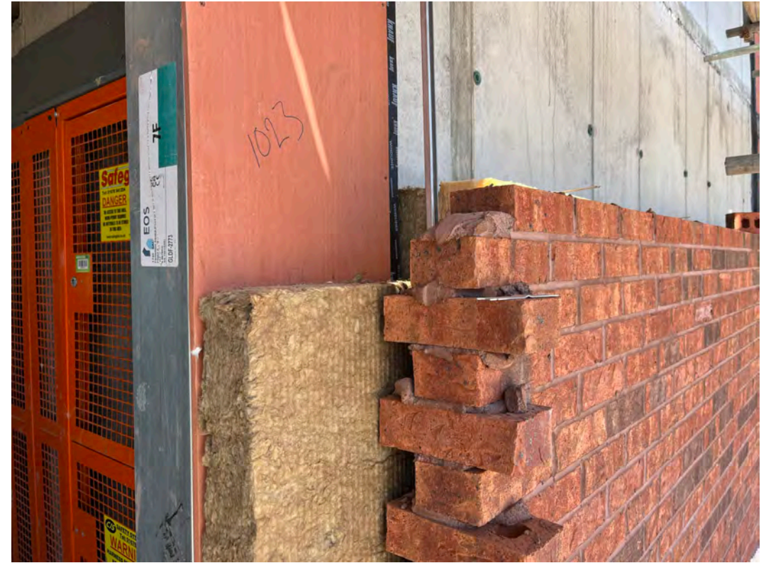
Block D – External brickwork and insulation ongoing
