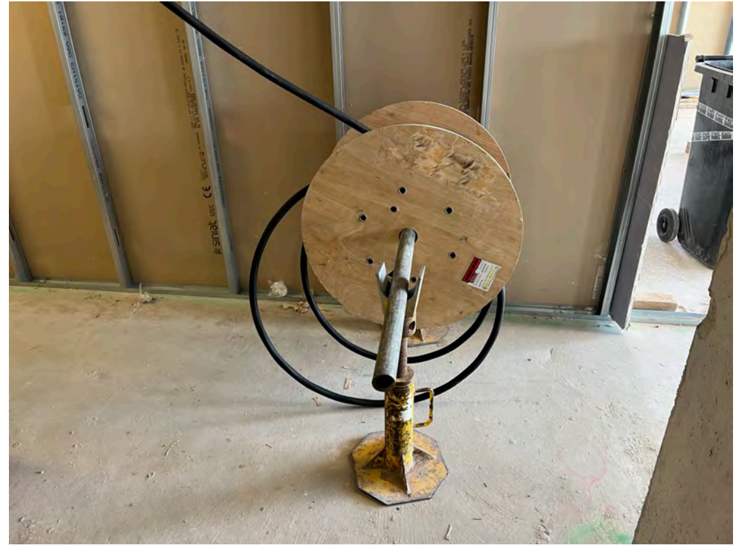
Sub-main installation ongoing to all levels
