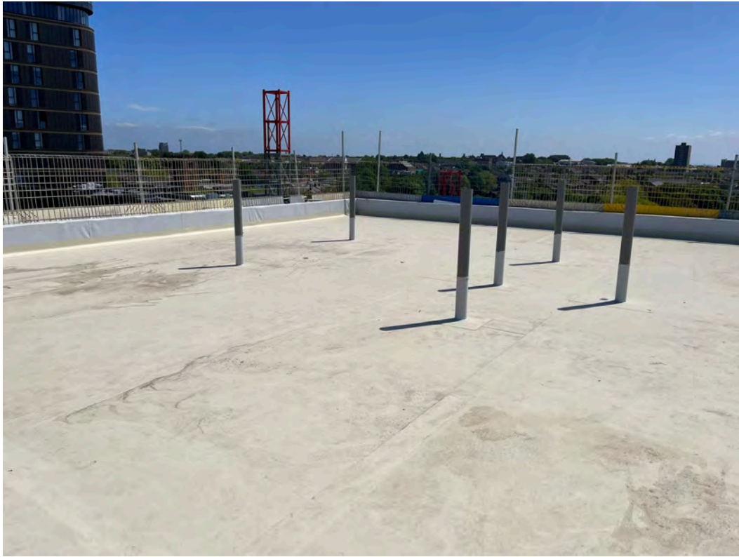
Block D Section A – Roof
