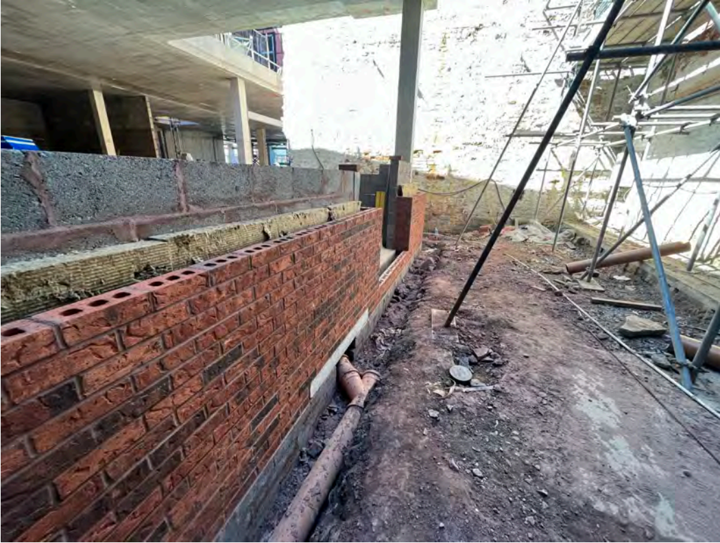
Ground floor external brickwork ongoing
