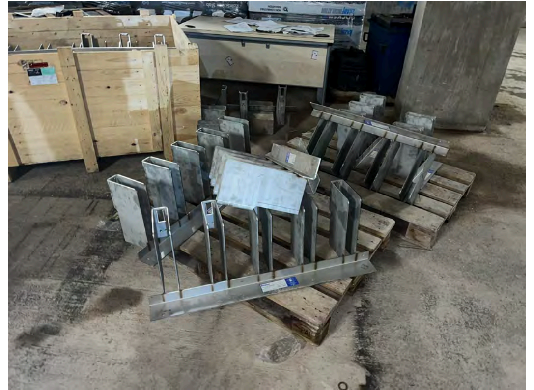
Materials on-site: Masonry support brackets
