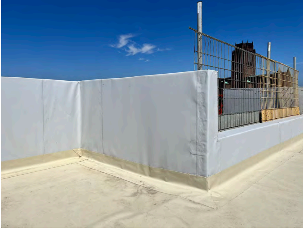
Block D Section A – Single ply membrane Installation
