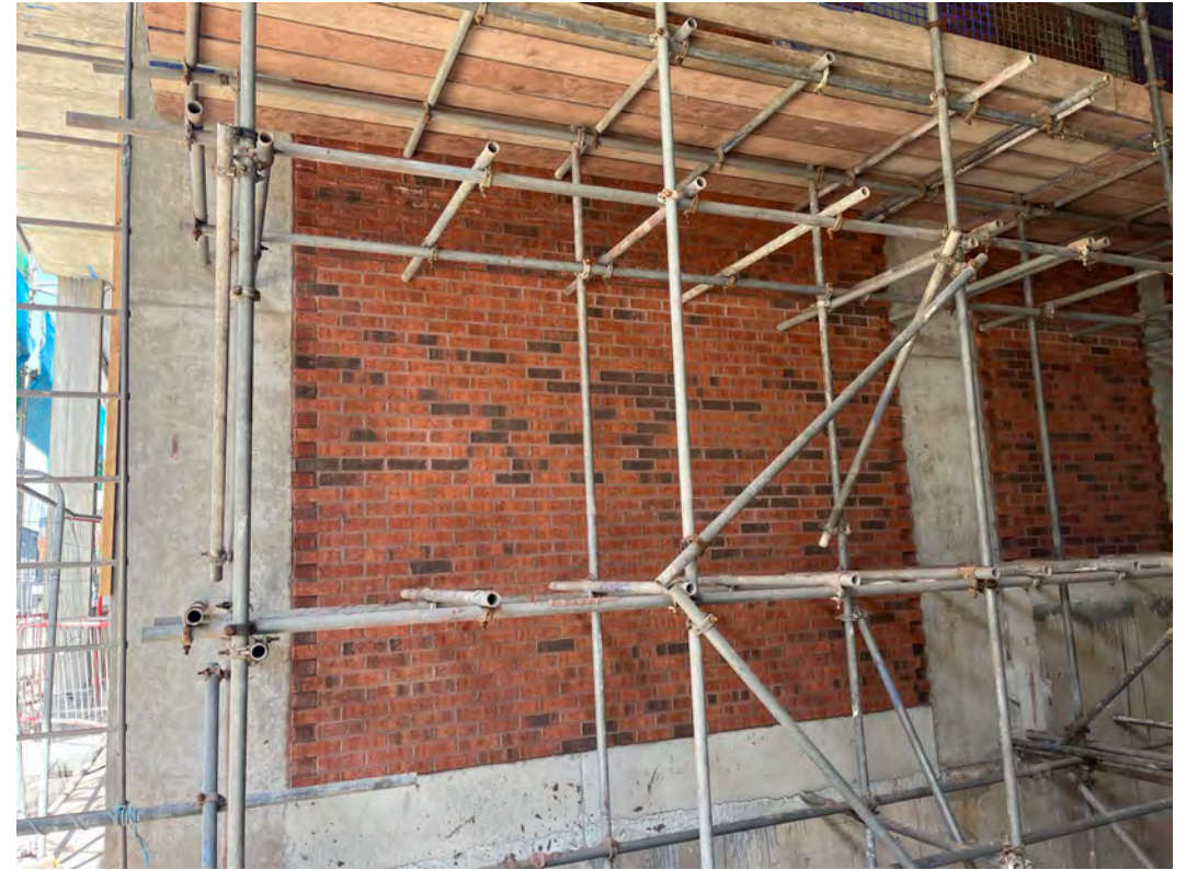
Ground Floor brickwork ongoing
