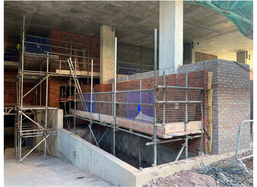
Ground floor brickwork walls
