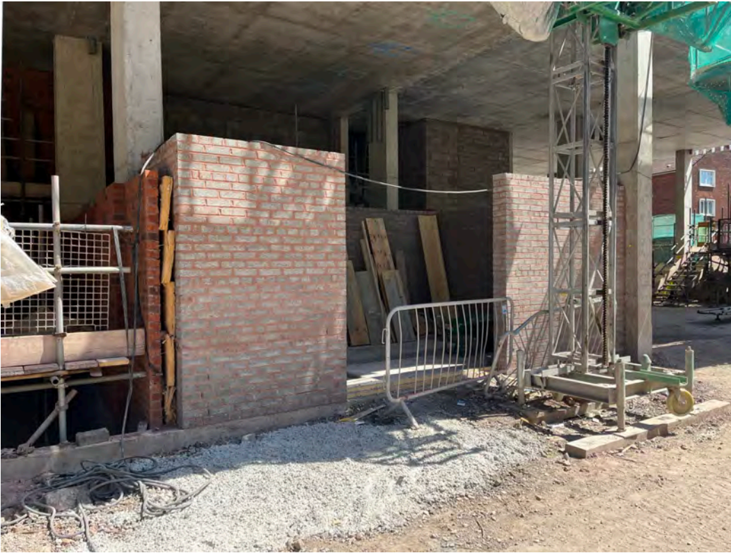
Sub-station construction ongoing
