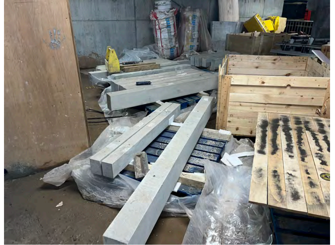
Materials on-site: Lintels
