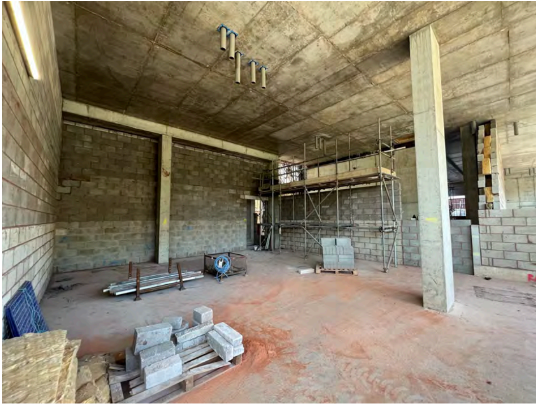
Ground Floor Internal blockwork ongoing
