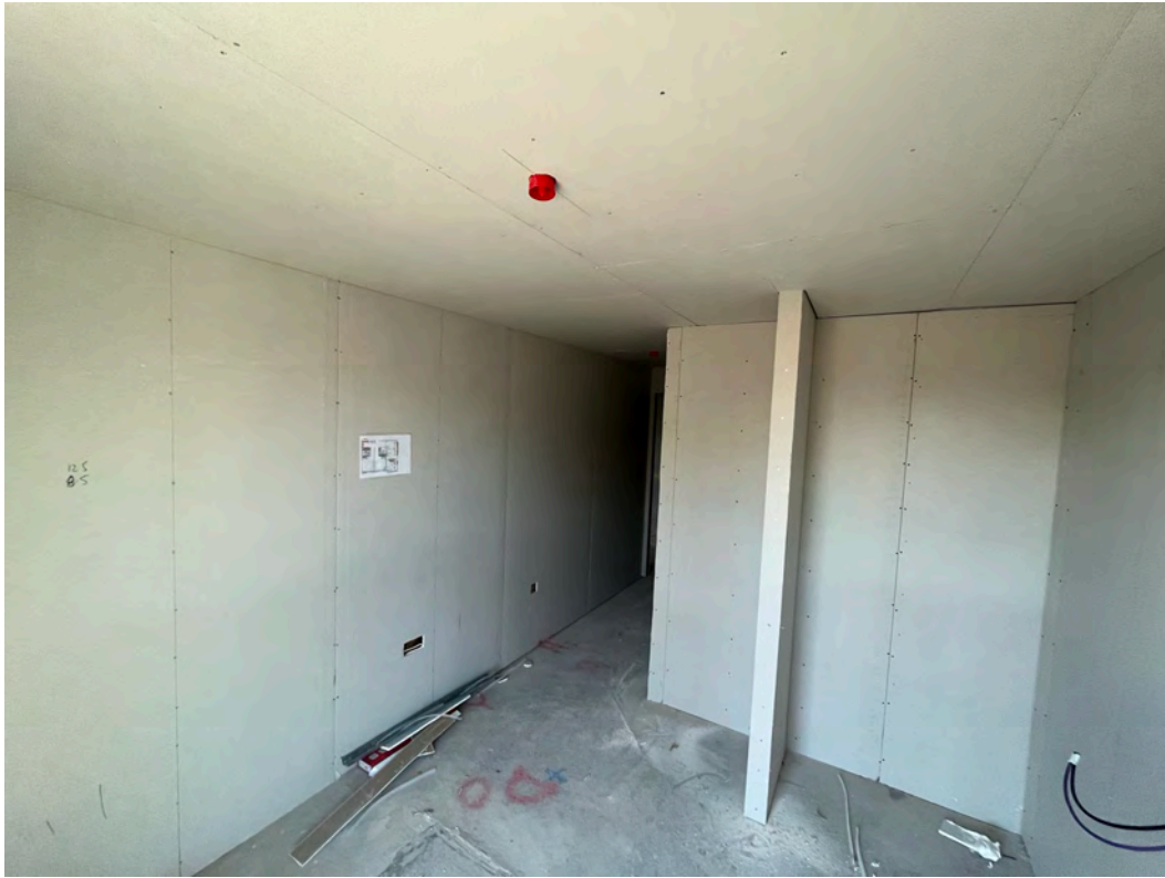
2 nd side boarding ongoing
