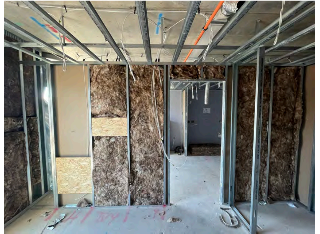
Insulation and pattress installation ongoing
