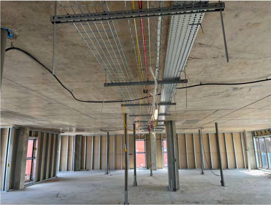
1 st fix electrical containment installation ongoing
