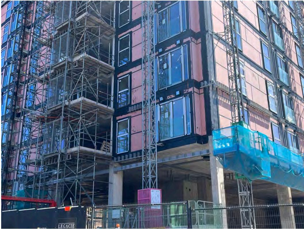
Block D Section A – Window units
