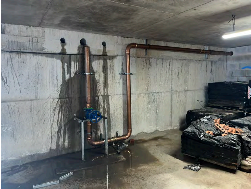
Main water distribution pipe installed
