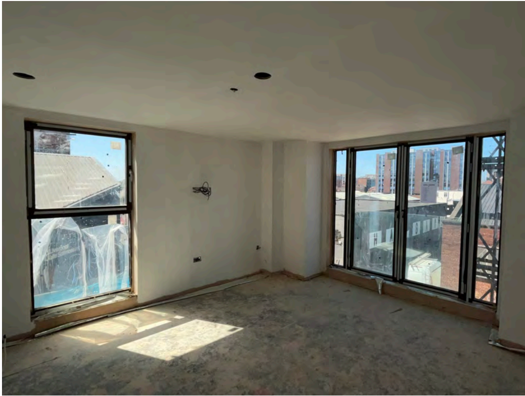
Mistcoat application to walls and ceiling ongoing
