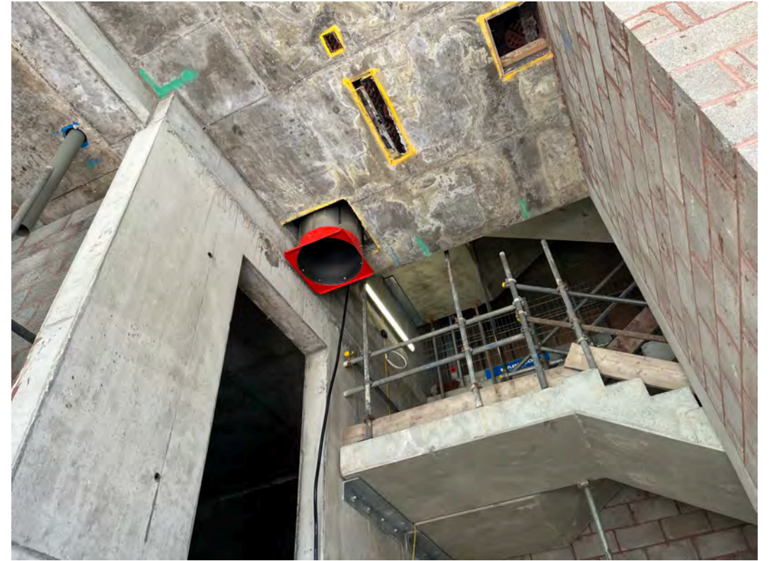
Bin chute installation has commenced
