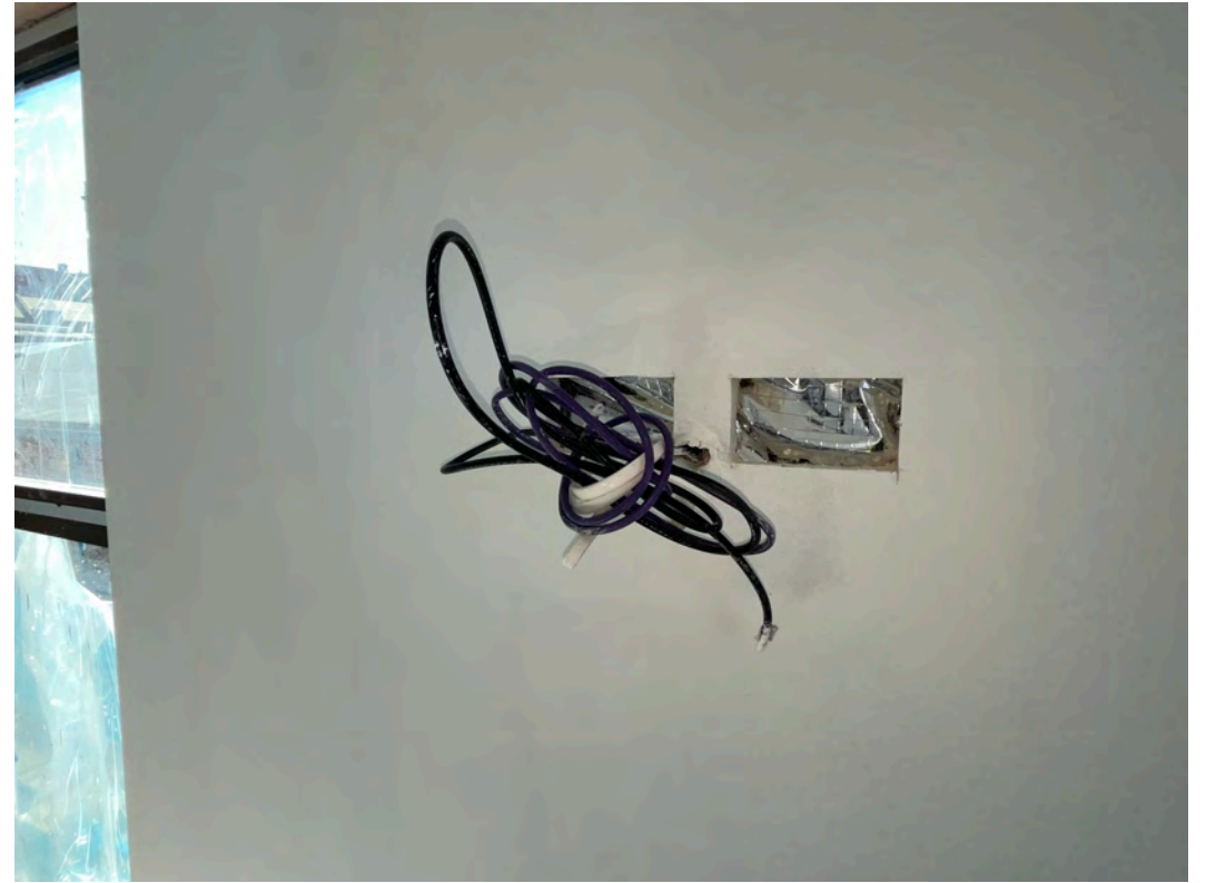
1 st fix electrical installation ongoing
