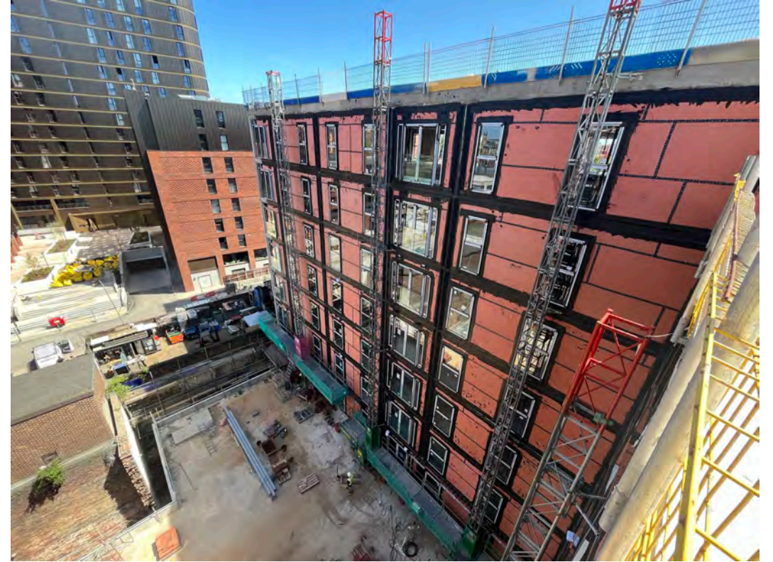
Block D Section B – SFS & Weatherboarding Installation
