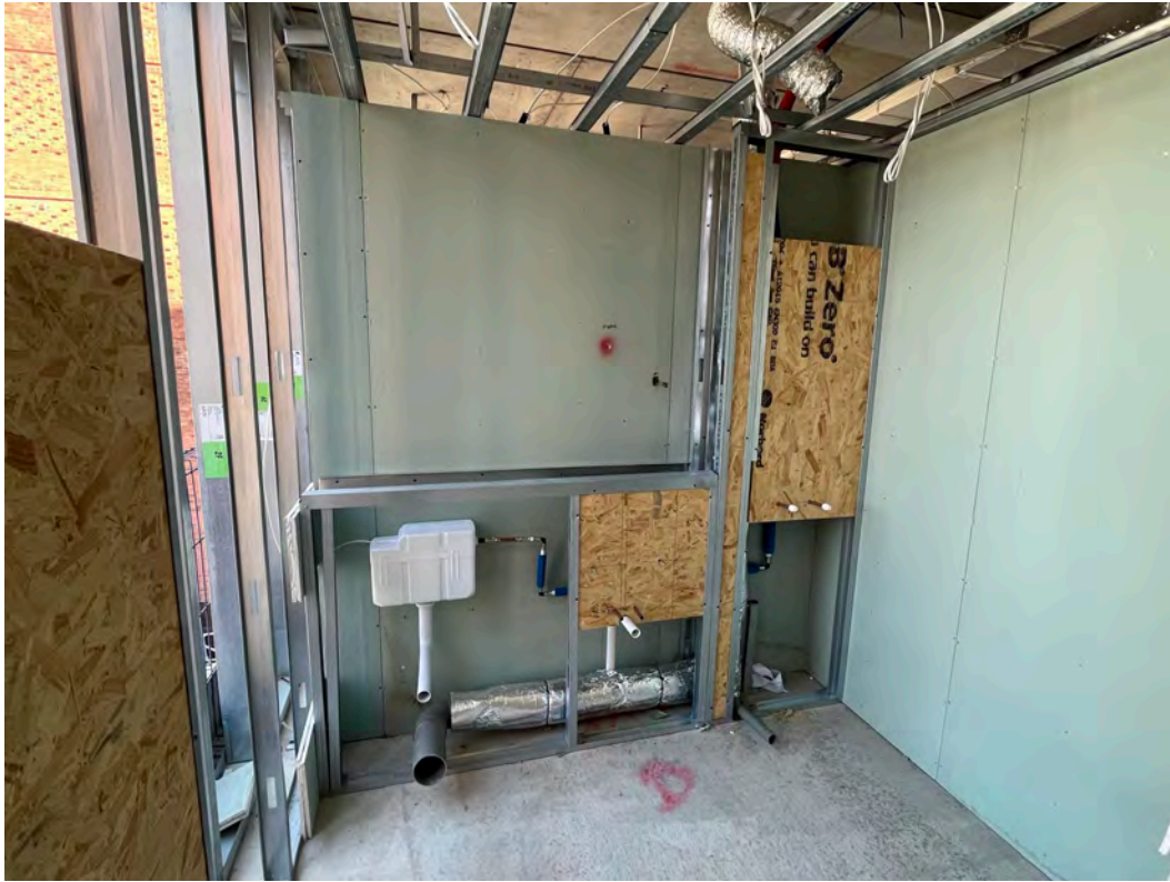
Formation of IPS and patress installation ongoing
