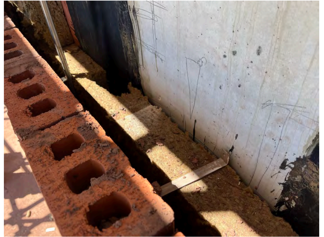
Block D – External brickwork and insulation ongoing
