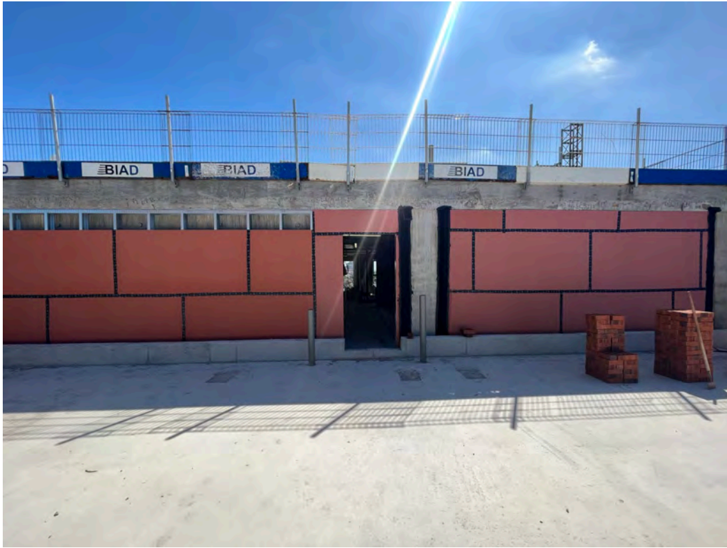
Block D – SFS & Weatherboarding Installation
