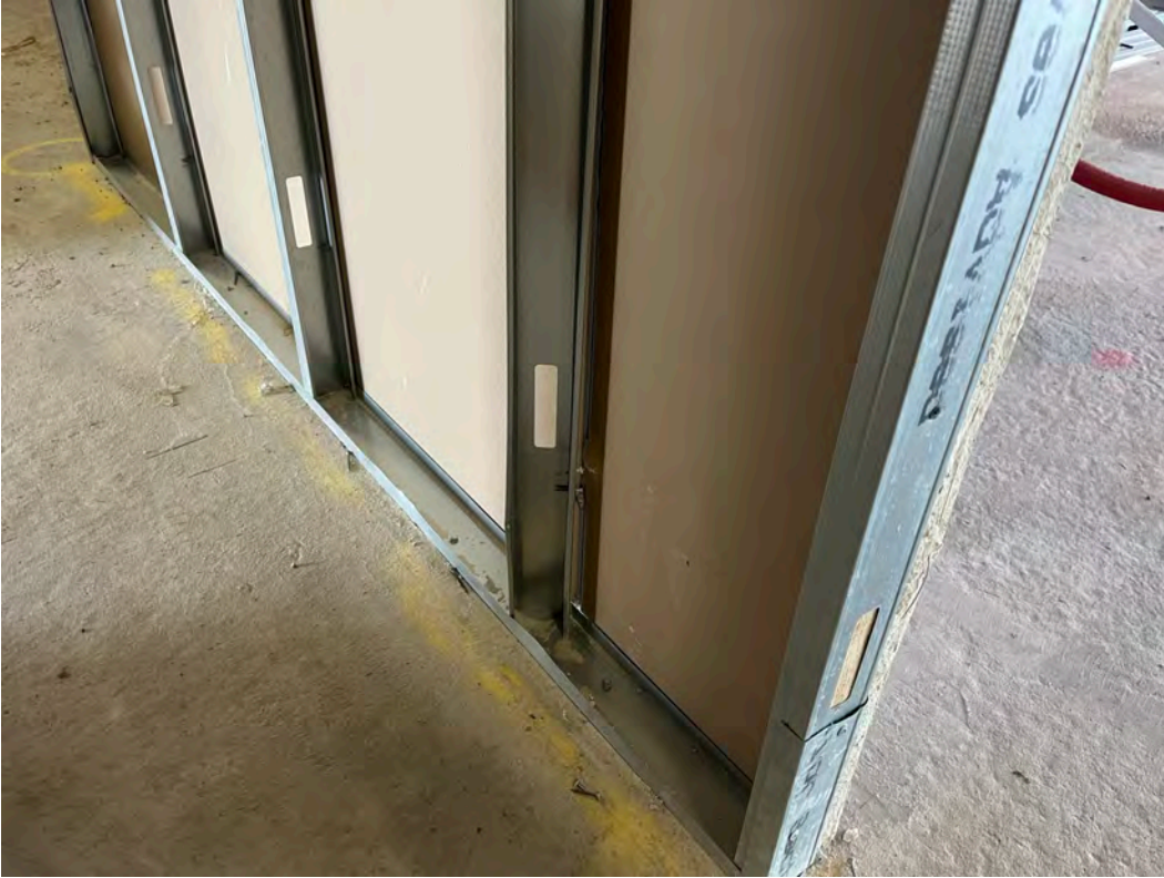
1 st side boarding ongoing
