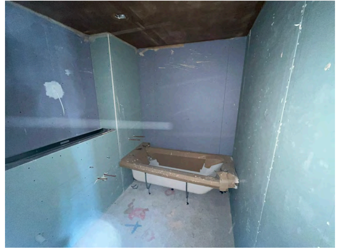
2 nd side boarding and sanitaryware installation ongoing
