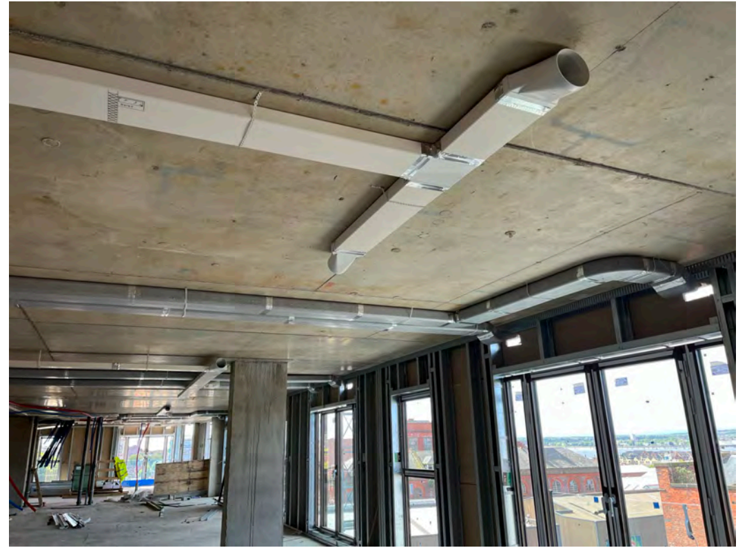
1 st fix mechanical ducting installation ongoing
