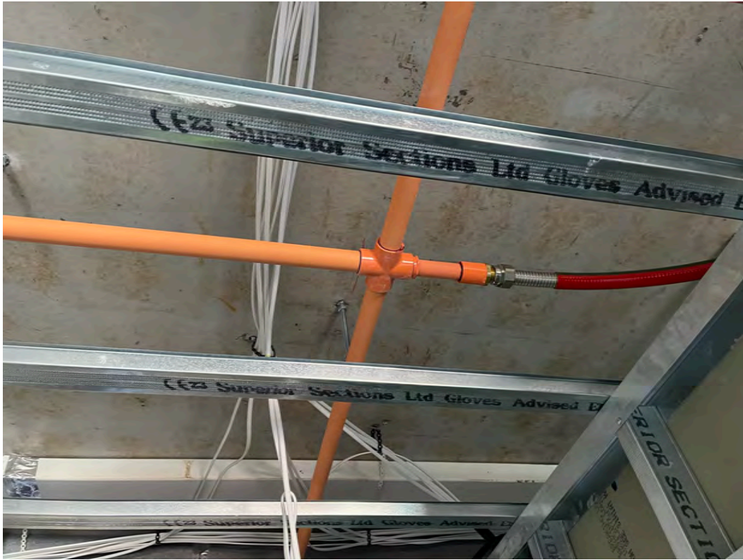
Sprinkler system installation ongoing
