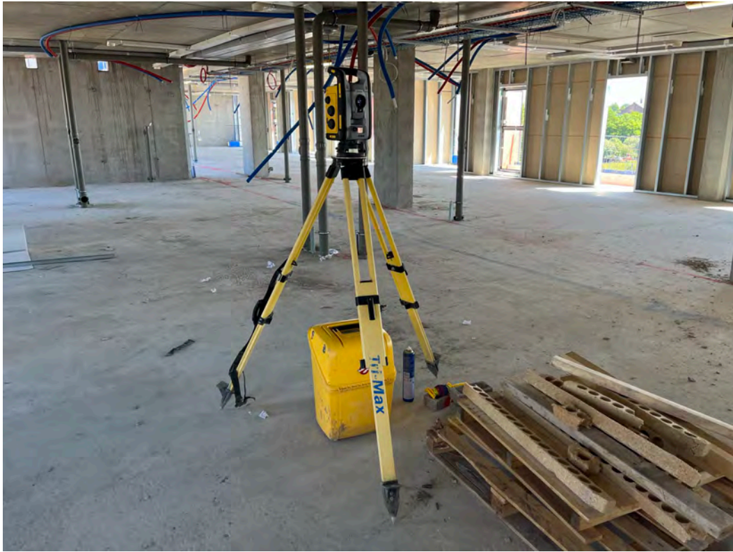
Apartment setting out ongoing
