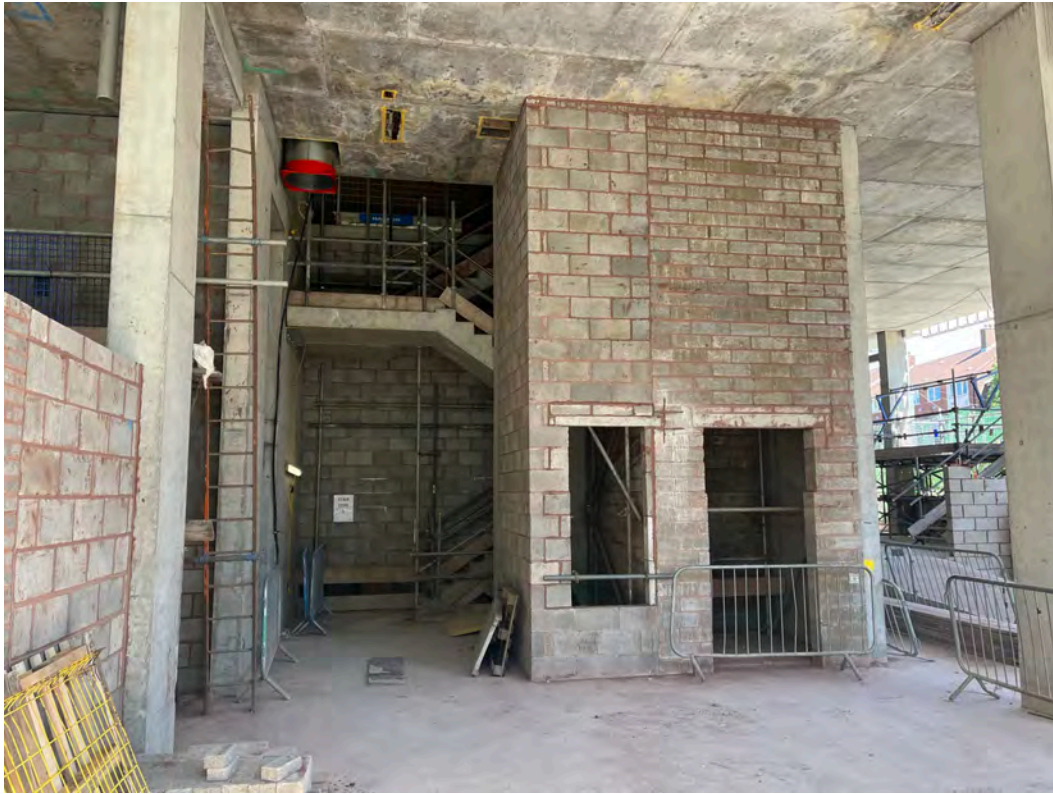
Lift shaft construction ongoing
