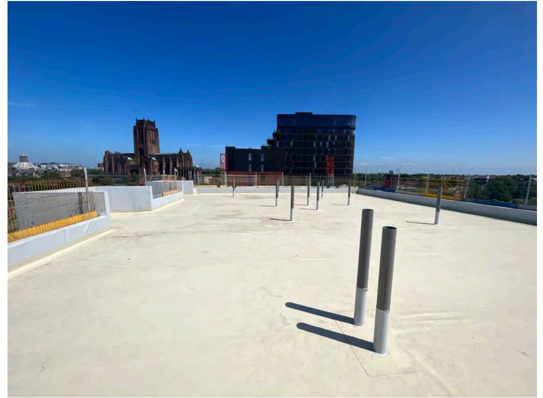
Block D Section A – Roof
