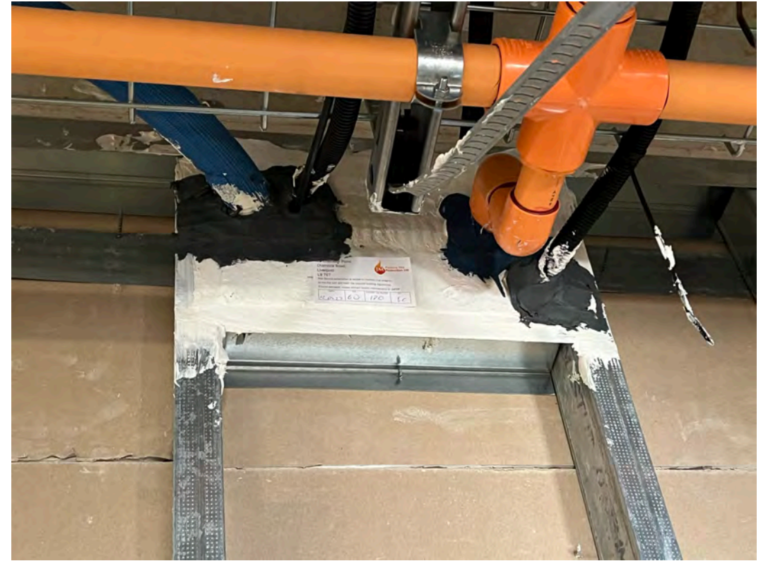
Fire stopping installation ongoing
