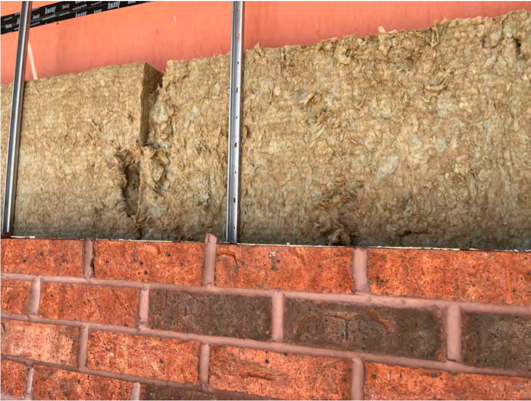
Block D – External brickwork and insulation ongoing
