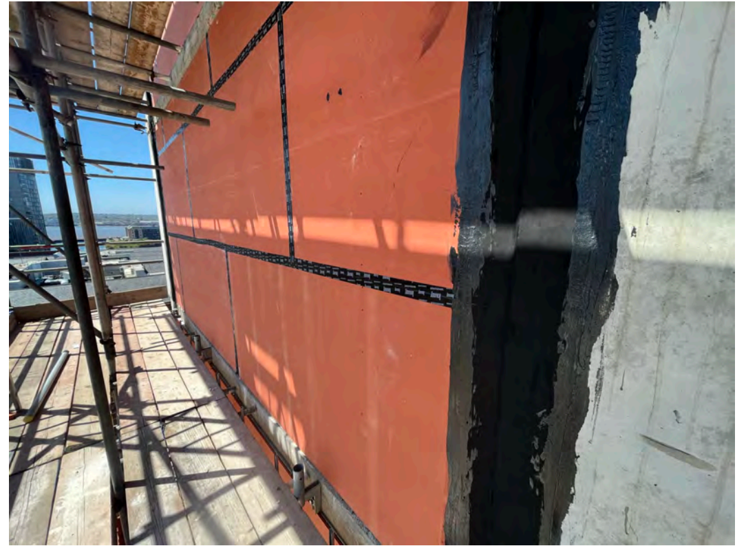
Block D – Weatherboarding and waterproofing Installation
