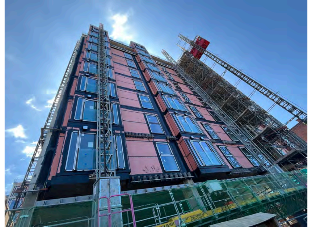
Block D Section B – Viewed from site compound
