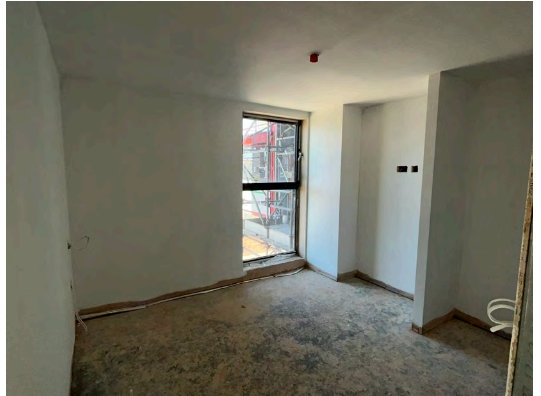
Mistcoat application to walls and ceiling ongoing
