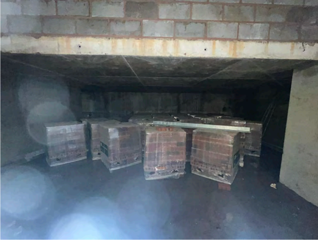
Materials on-site: Brick
