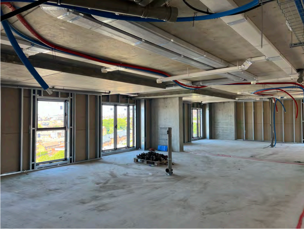
Apartment 1 st fix mechanical installation ongoing
