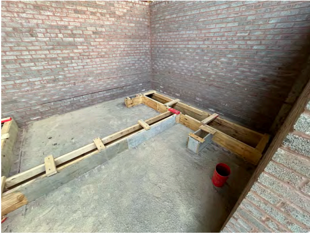
Ductwork channels formed to substation
