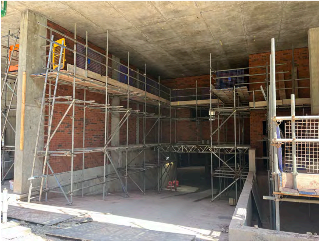
Ground Floor brickwork ongoing
