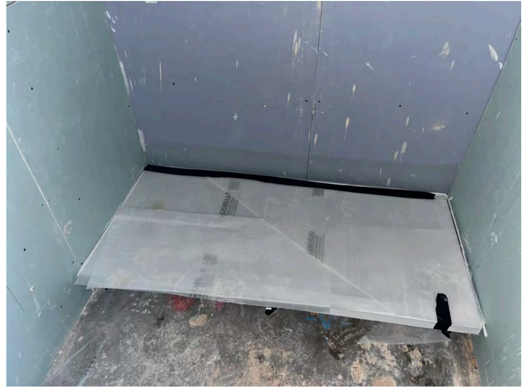
Aanitaryware installation ongoing
