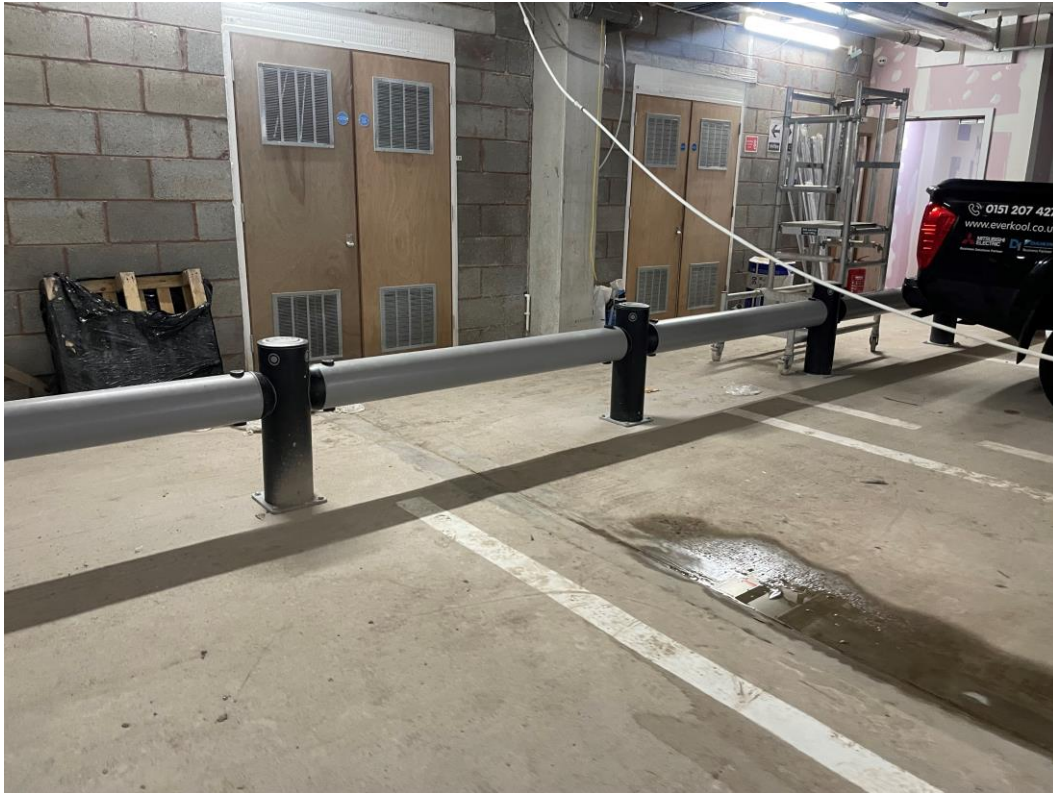
A-Safe vehicle barriers installed
