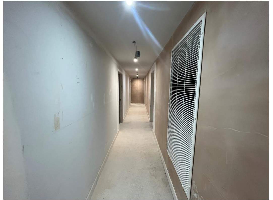
Circulation area finishes
