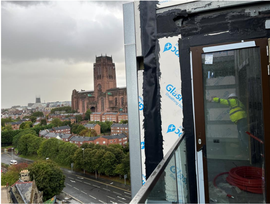
Liquid water proofing ongoing
