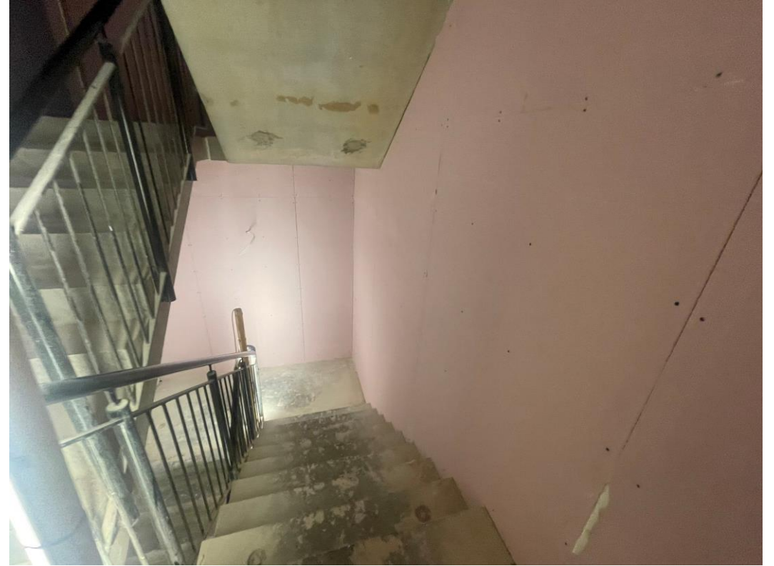
Boarding to staircase areas
