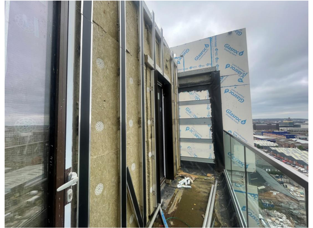
Insulation installed
