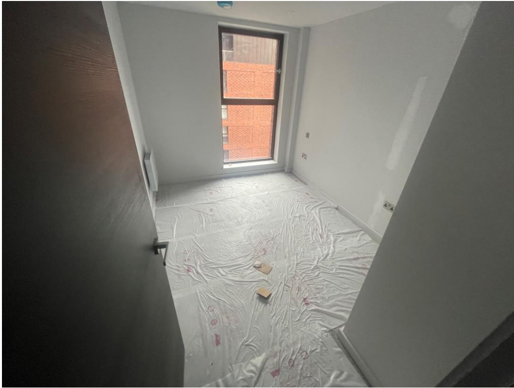
Bedroom carpets installed to upper levels
