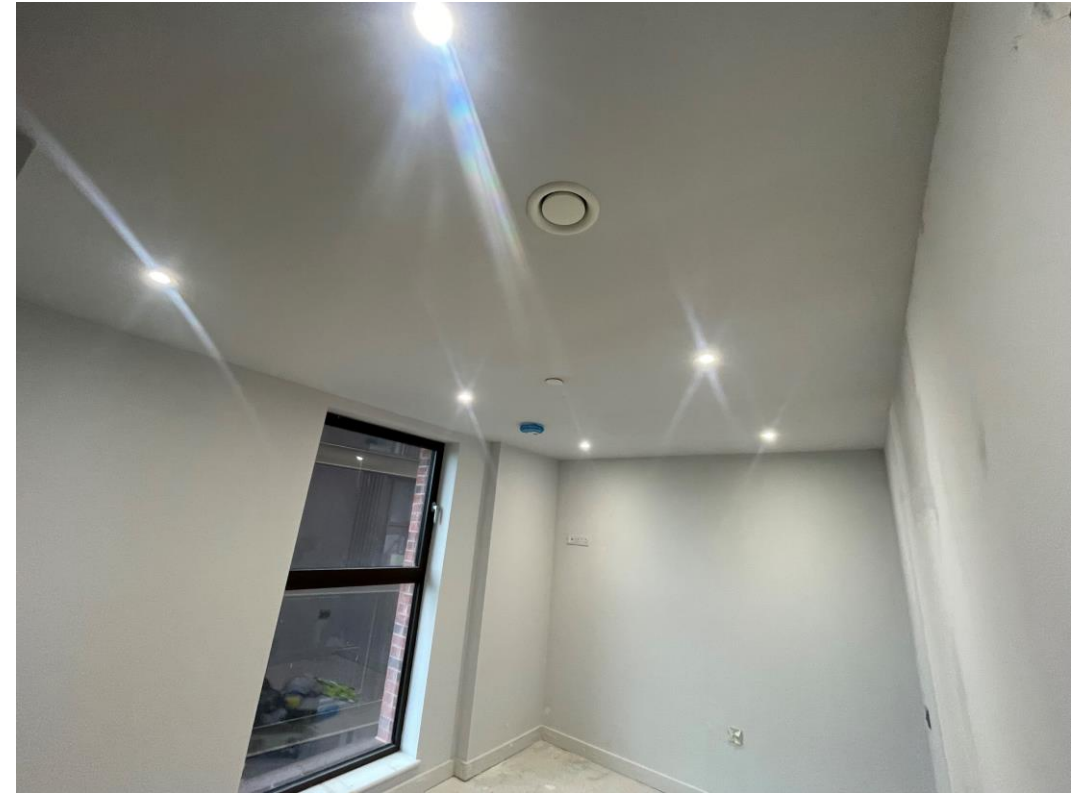
2 nd Coat decoration to bedroom wall & ceilings
