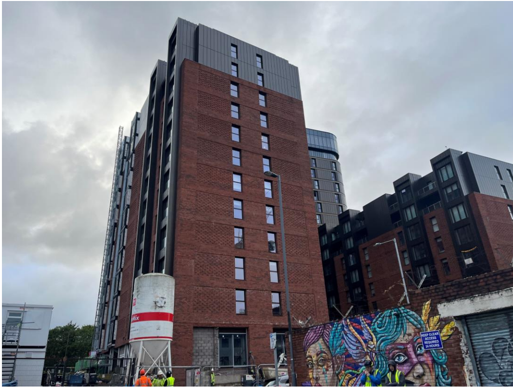
Block B – Viewed from Greenland Street
