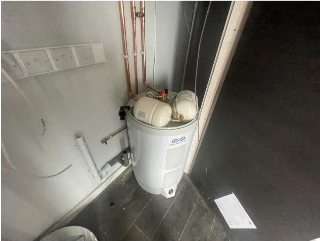
2 nd Fix M&E installation ongoing
