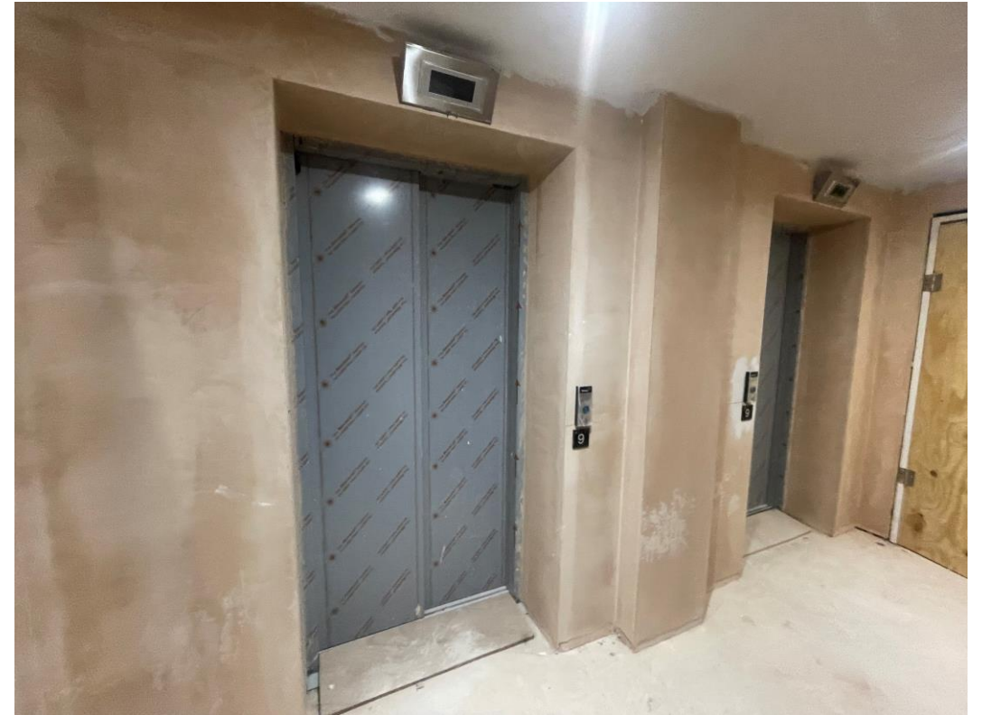
Lift lobby finishes ongoing
