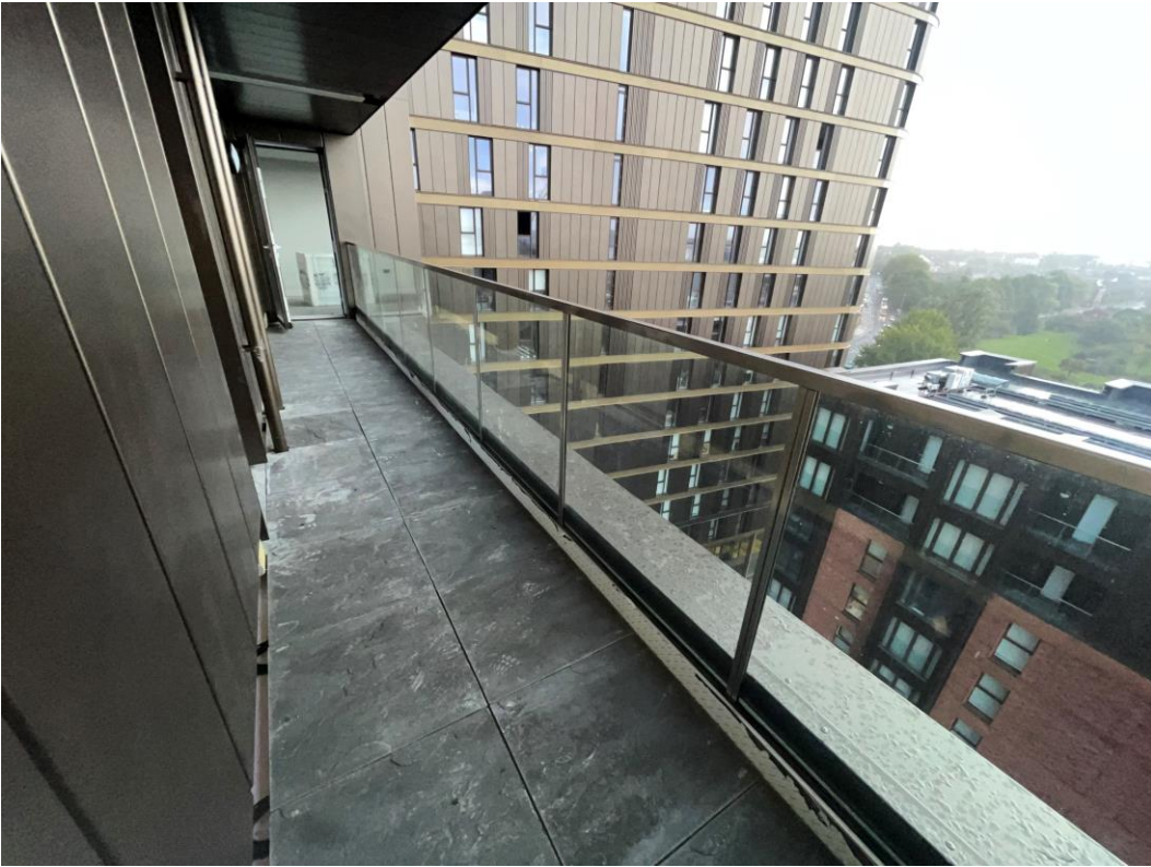
Glazed balustrade installed
