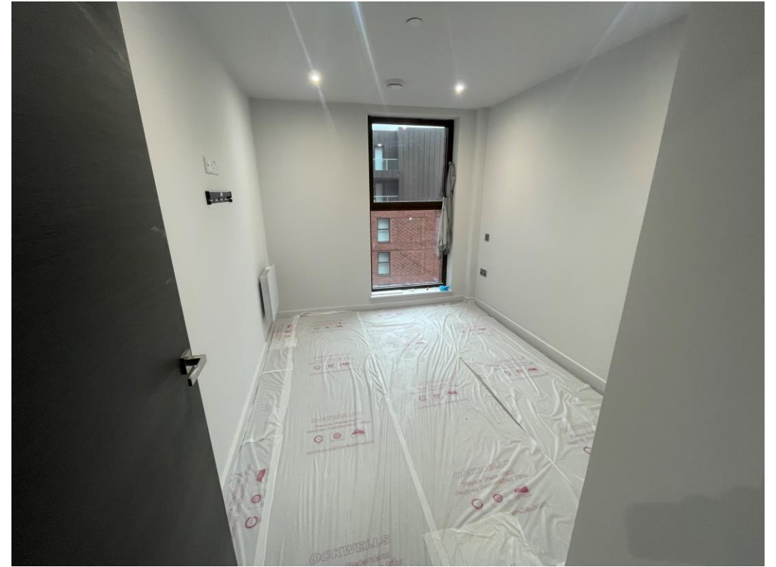
Bedroom carpets installed to upper levels
