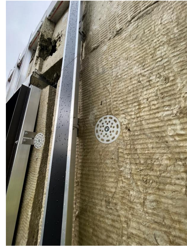
Cladding framework installation ongoing
