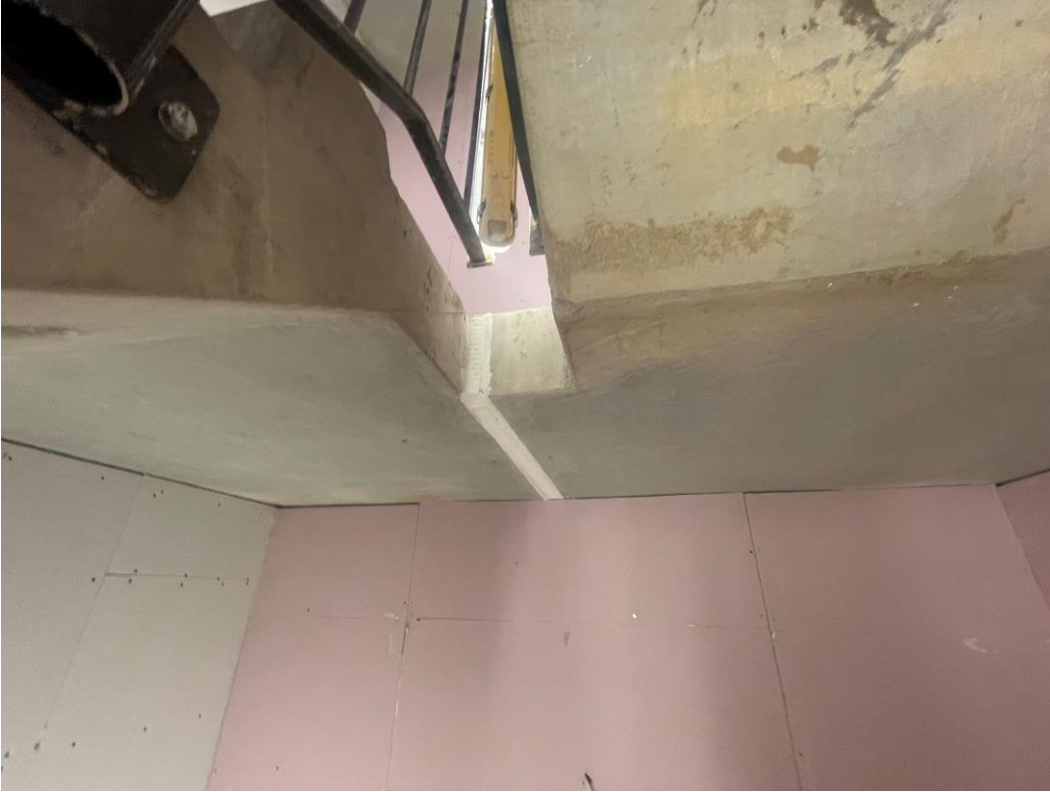
Staircase joint infill
