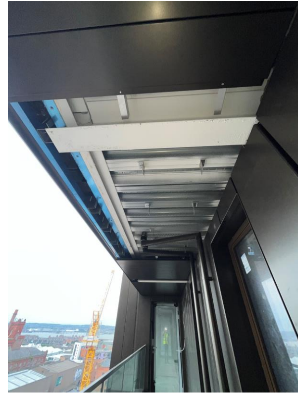
Soffit cladding installation ongoing
