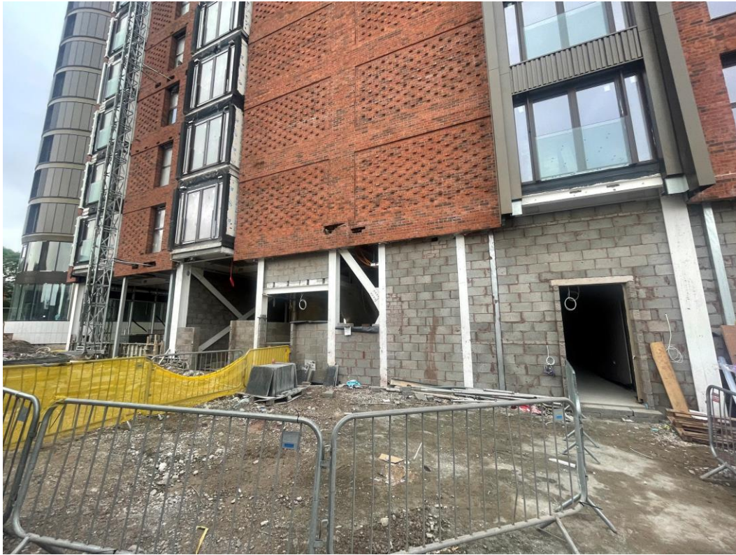
Block B – Forming of Block B entrance
