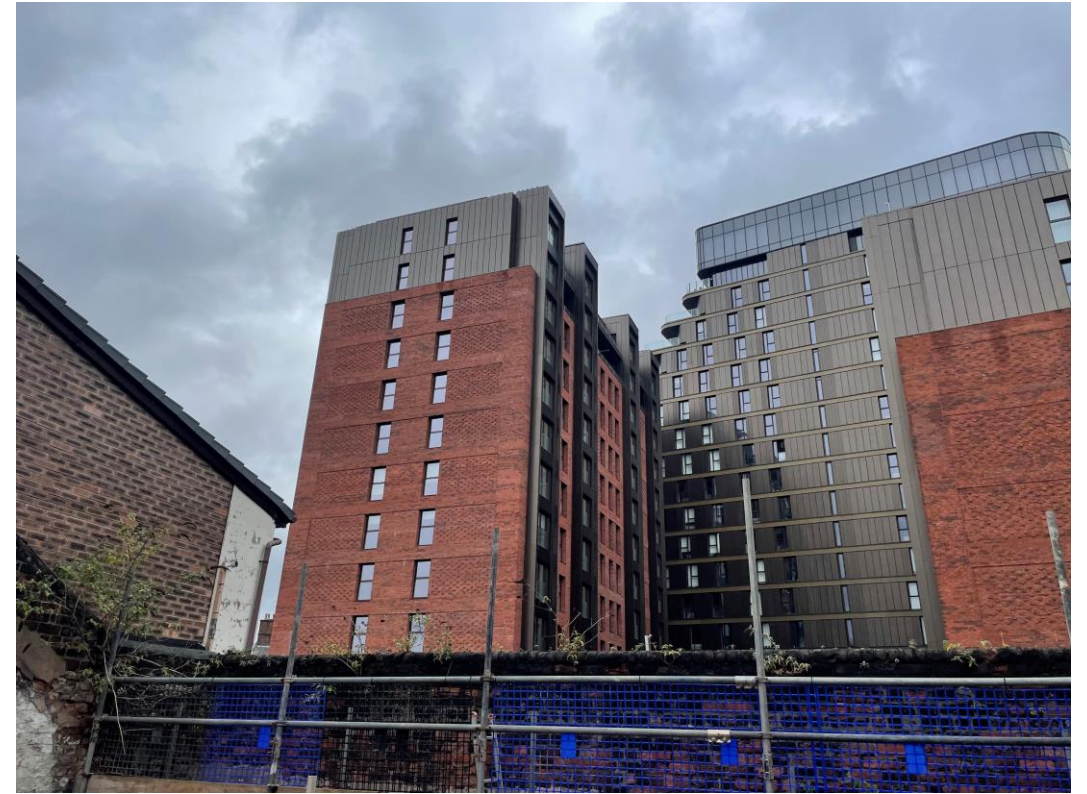
Block B – Viewed from Block D
