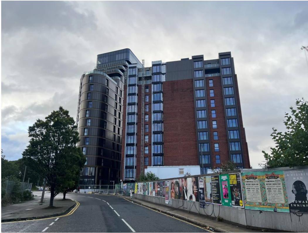
Block B – Brickwork & cladding installation
