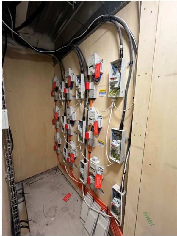
Electrical meters installed
