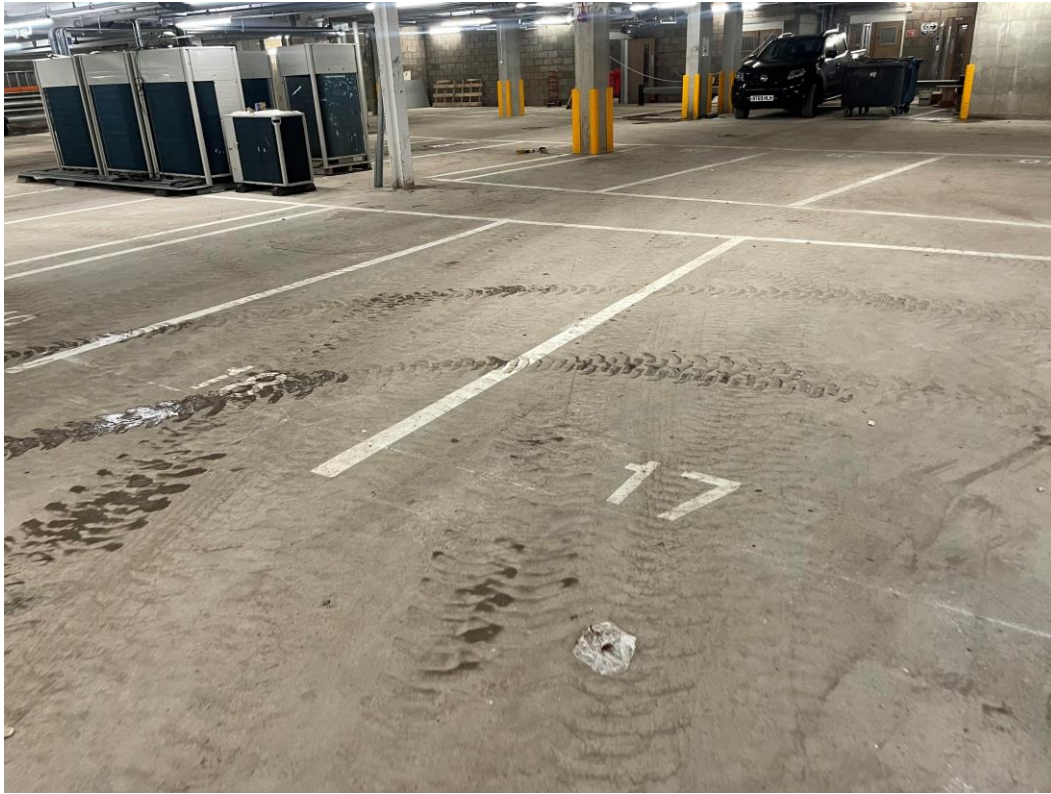
Road markings installed
