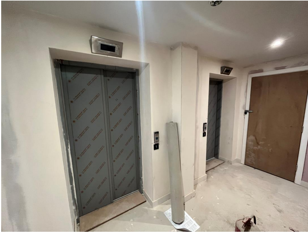
Lift area finishes
