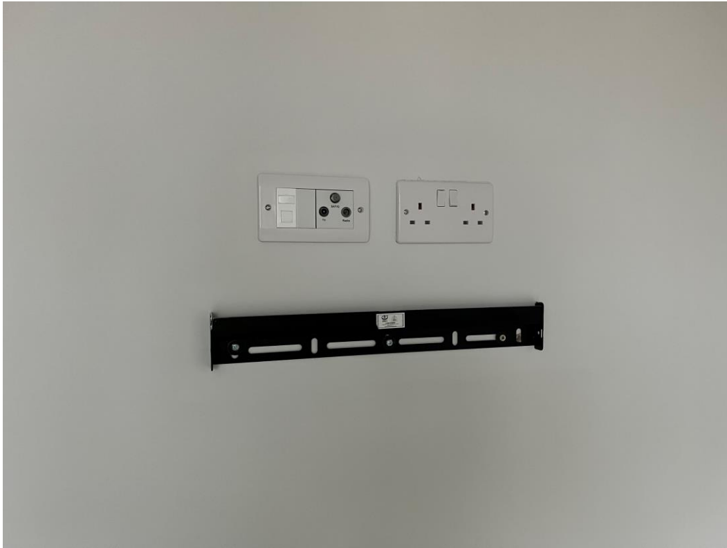
Tv bracket installed
