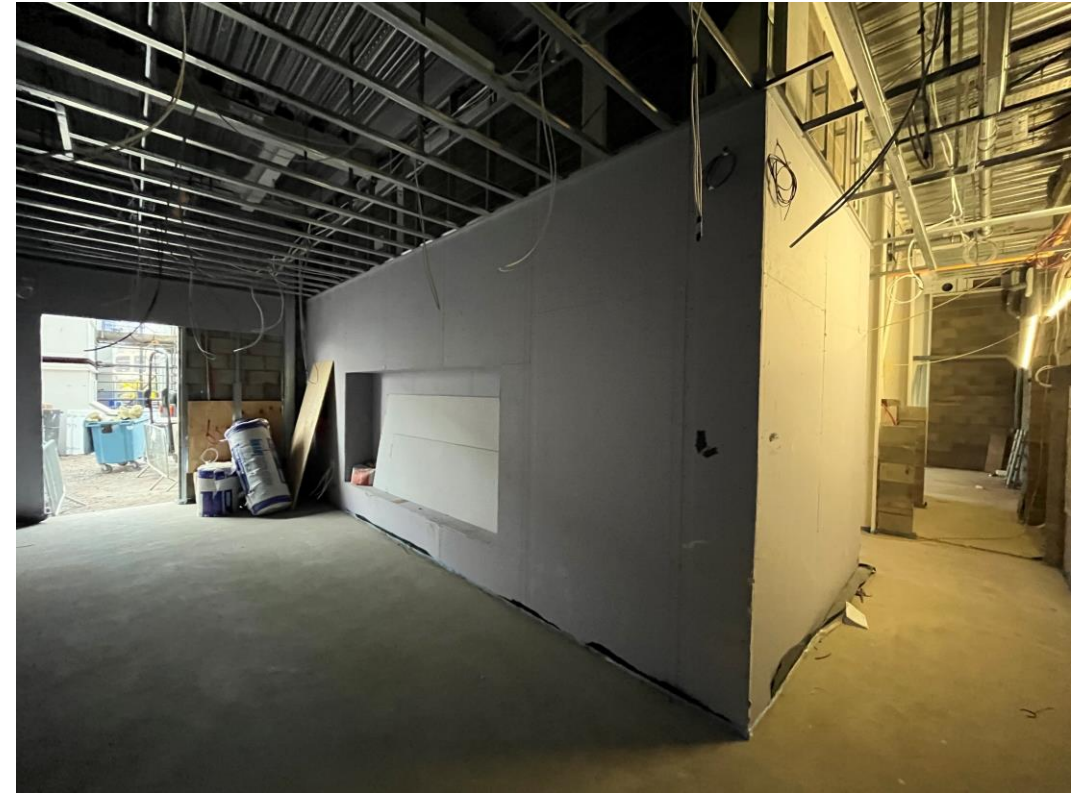
Plaster board installed
