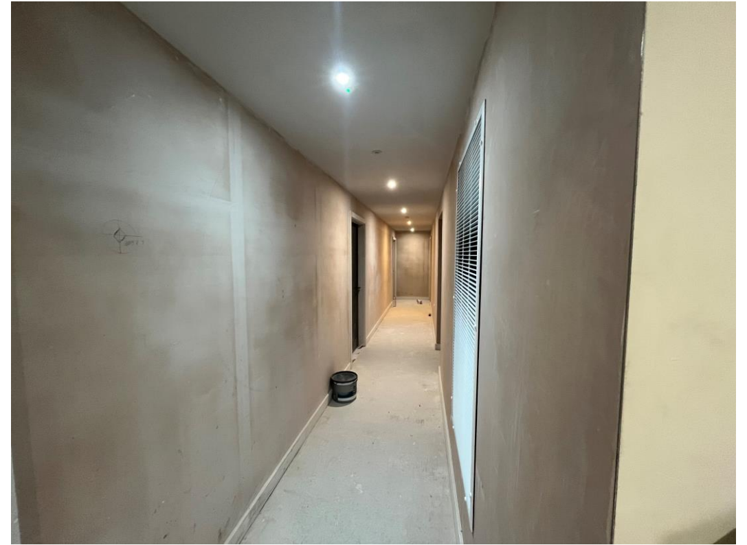
Circulation area finishes
