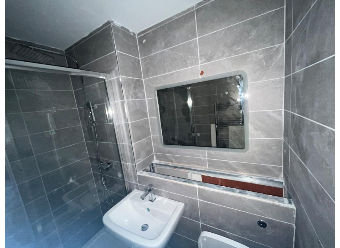
Bathroom mirror installed
