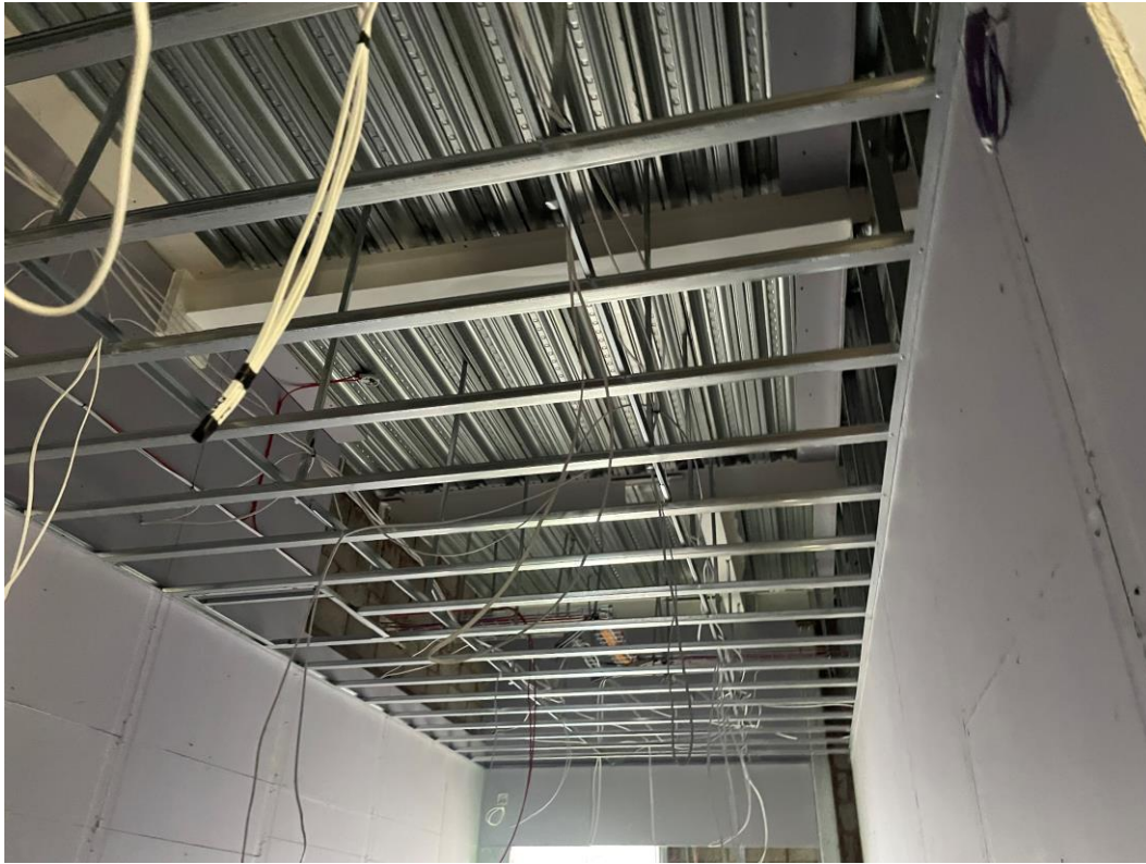
Ceiling grid installed
