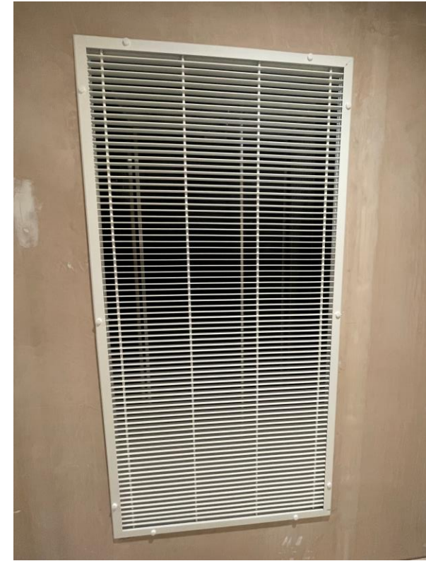
Ventilation covers installed
