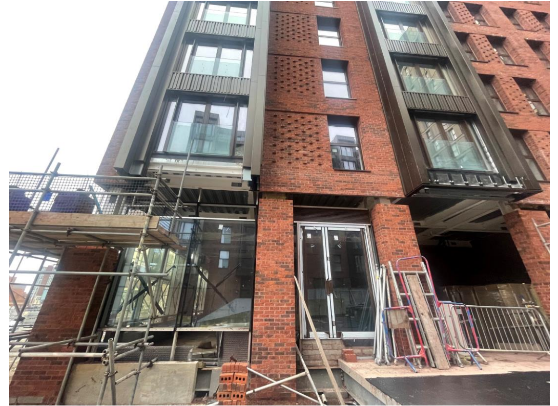
Block B – Window & Door Installation
