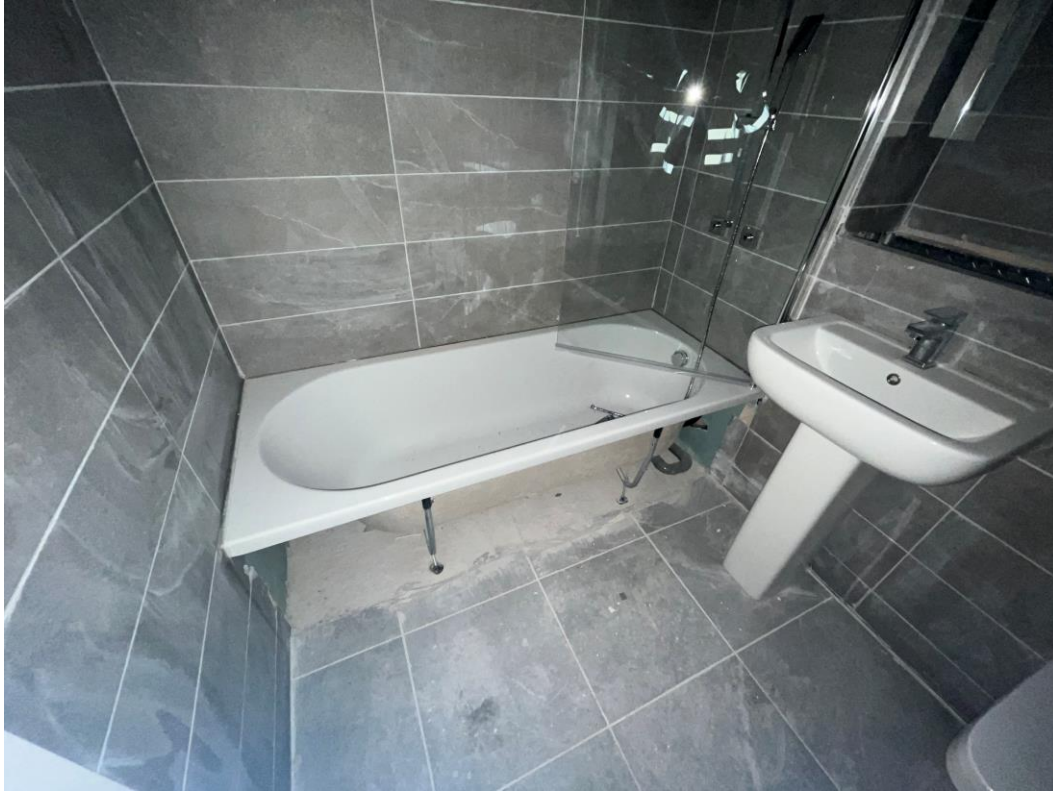
Bathroom appliances installed
