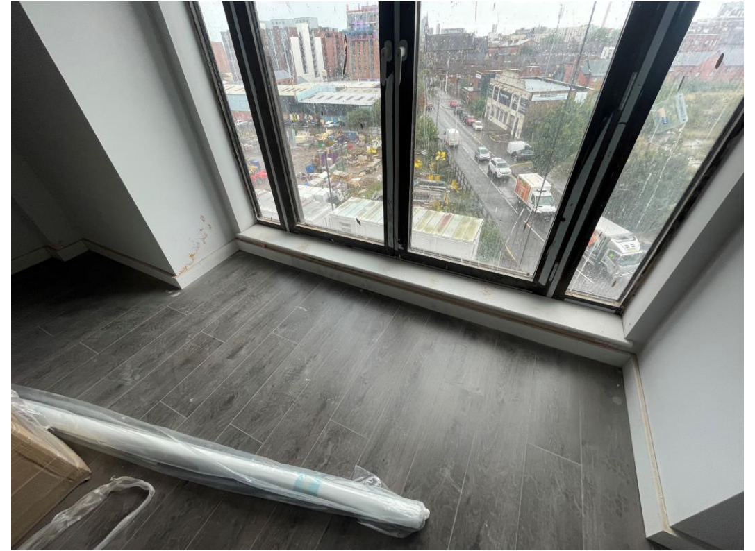
Window boards installed
