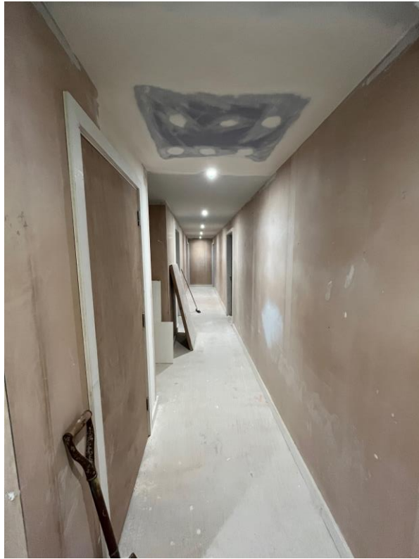
Circulation area finishes
