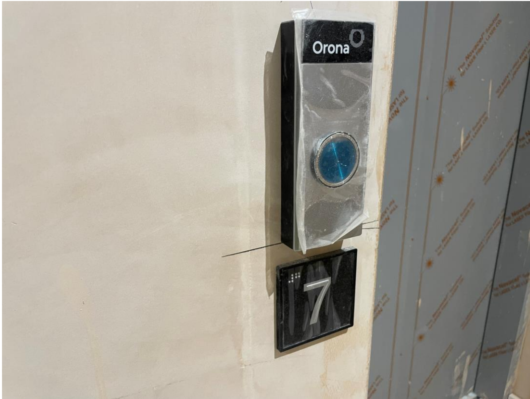
Lift level numbers installed
