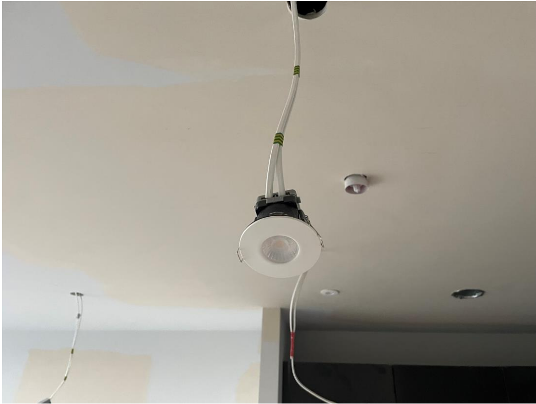
2 nd Fix M&E ongoing
