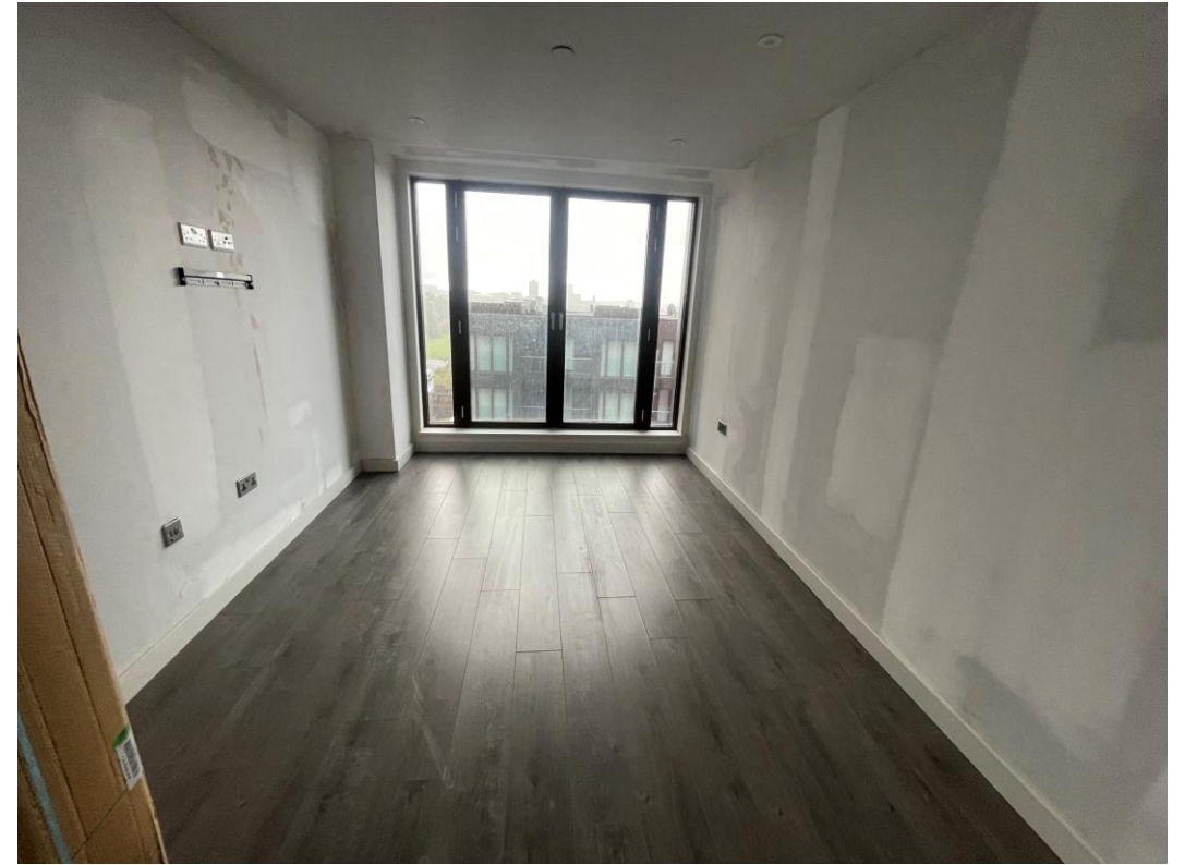
Lounge finishes ongoing
