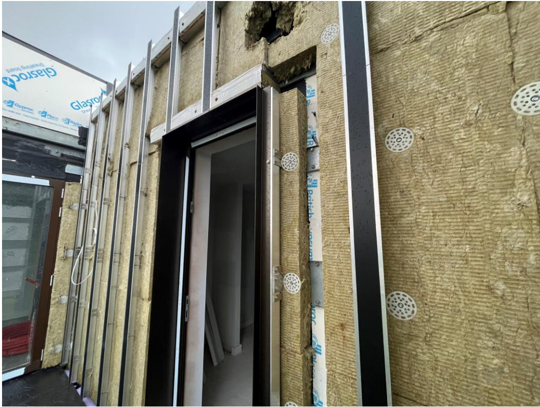
Insulation installed
