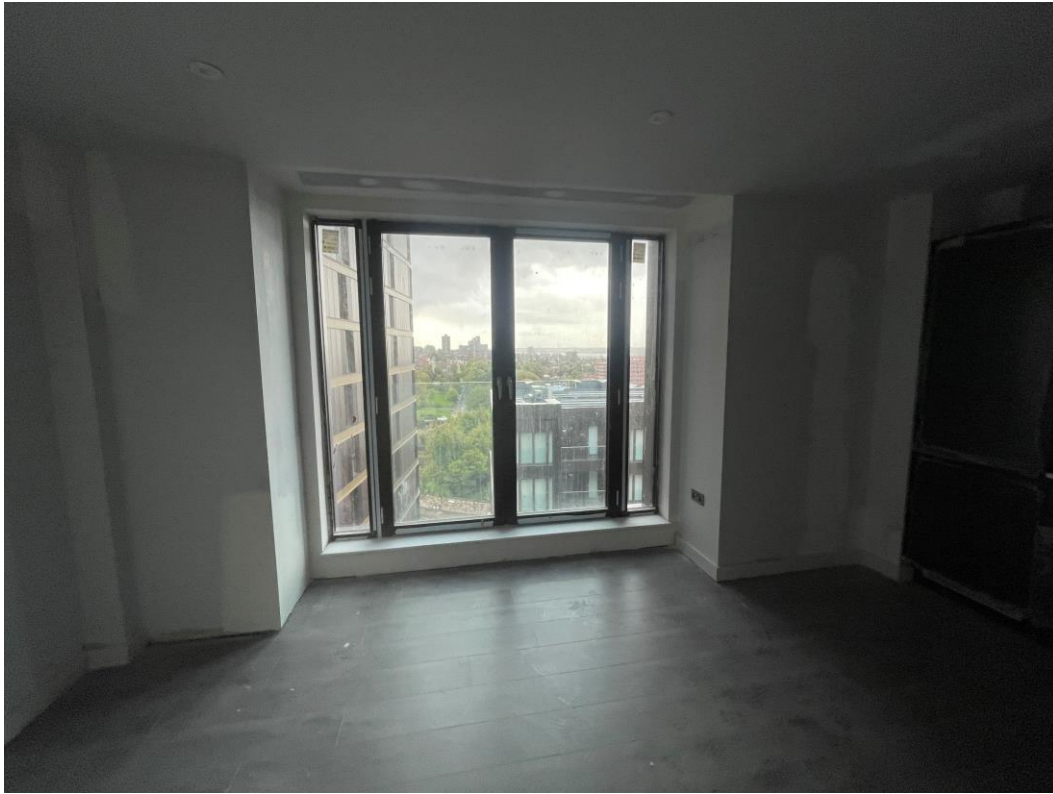
Lounge finishes ongoing
