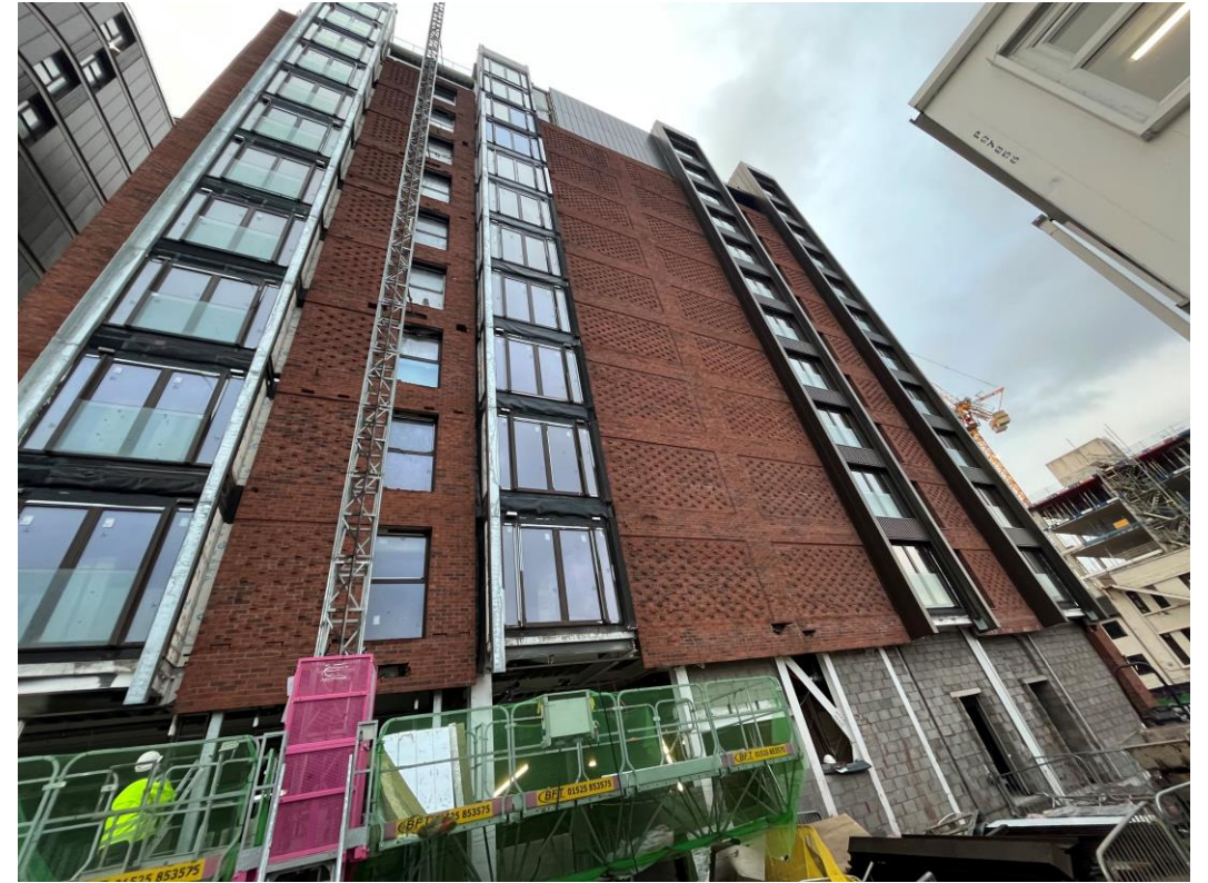
Block B – Brickwork & cladding installation
