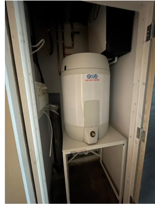
2 nd Fix M&E ongoing
