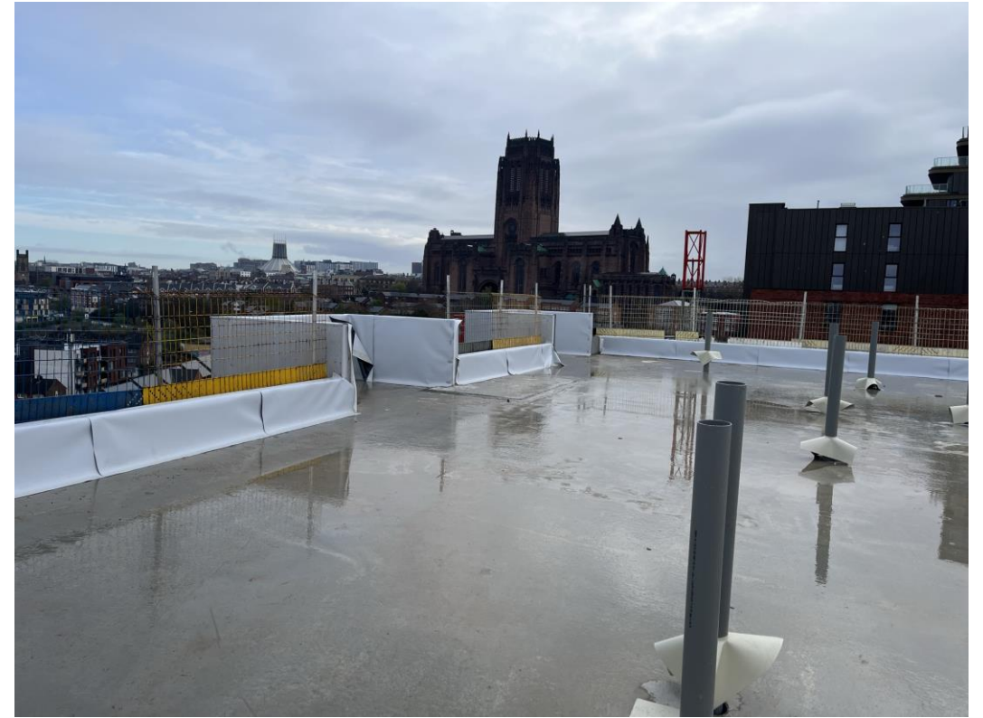
Block D Section A - Single ply membrane Installed to parapet walls
