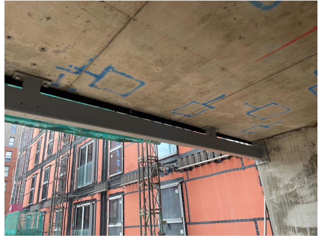
Block D – Curtain wall supports
