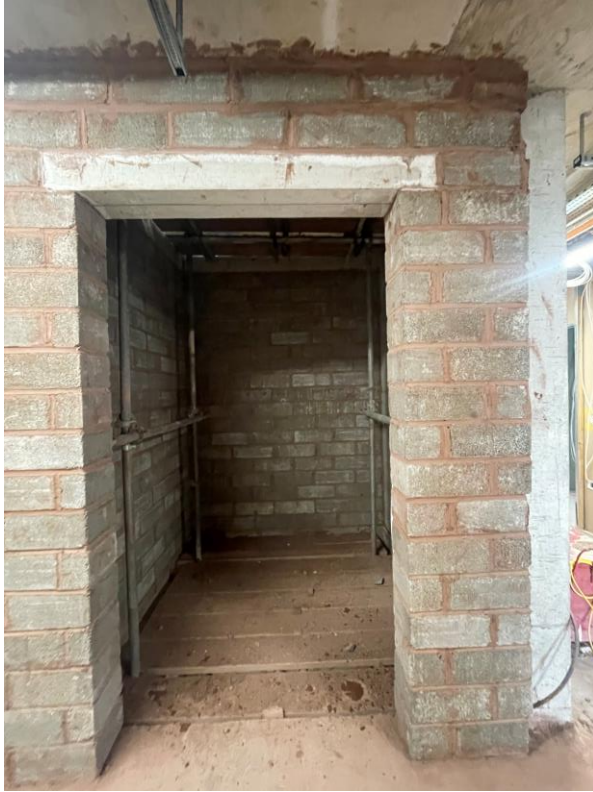
Lift shaft blockwork
