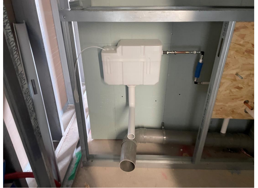
WC Cistern installation commenced
