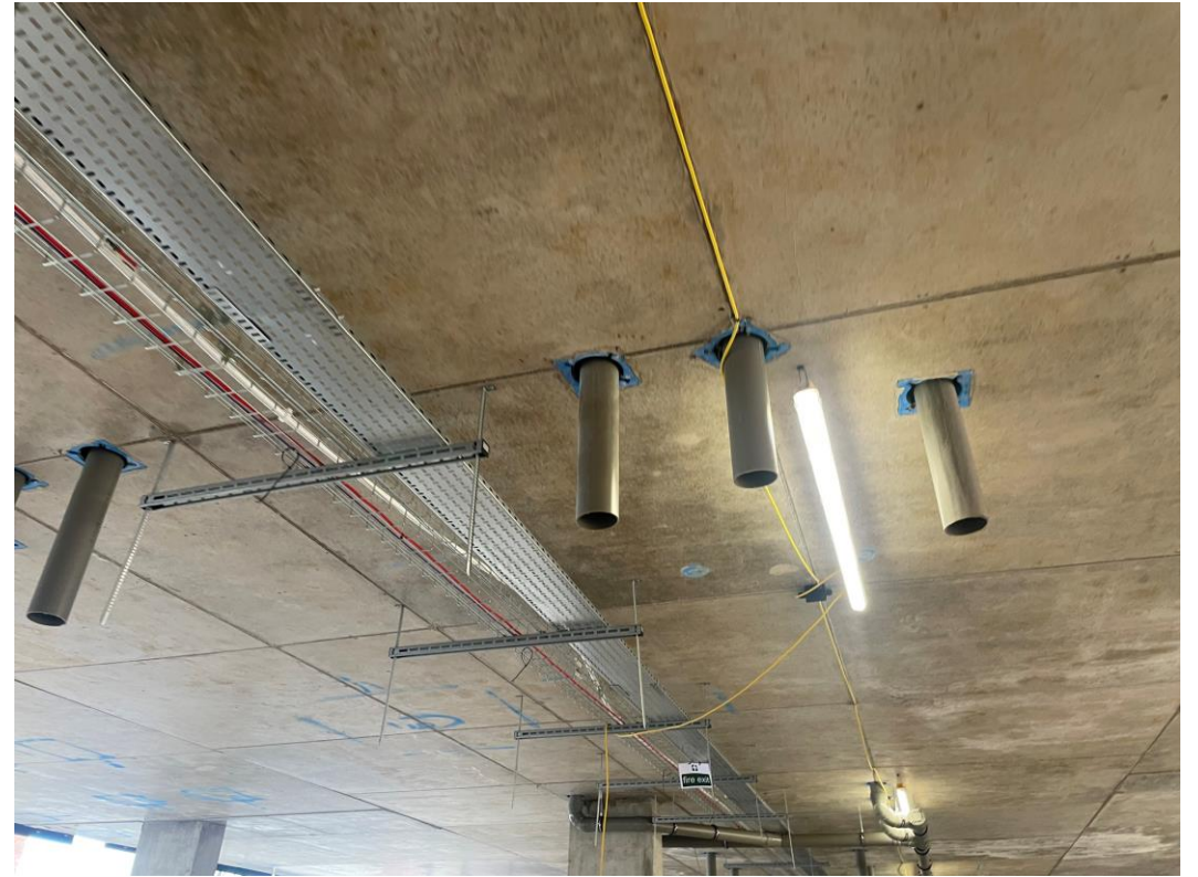
Apartment drainage ongoing
