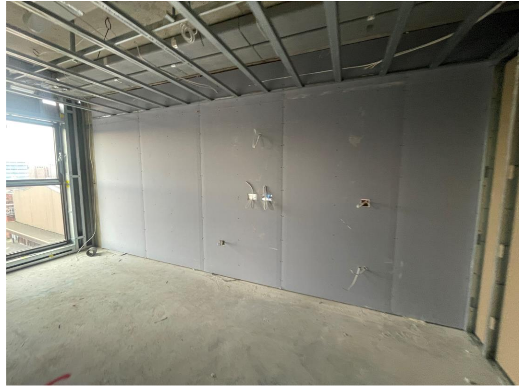
1 st fix Electrical installation ongoing
