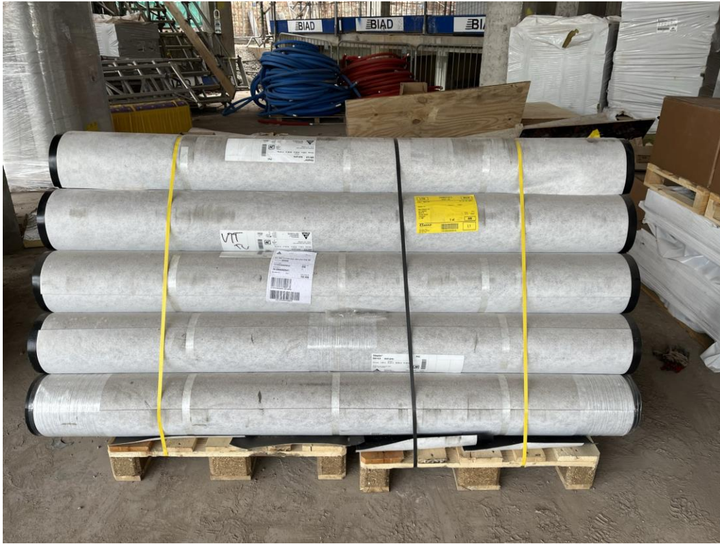
Single ply membrane stored onsite for installation
