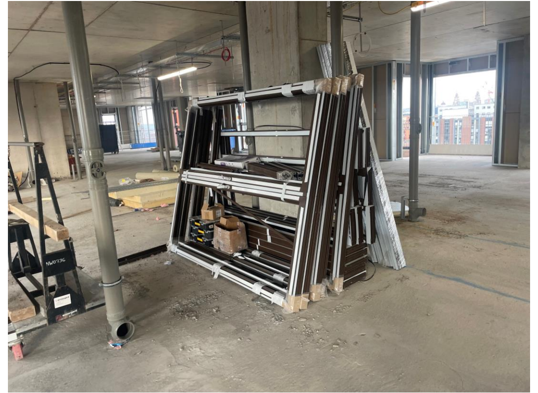
Window frames on site for installation
