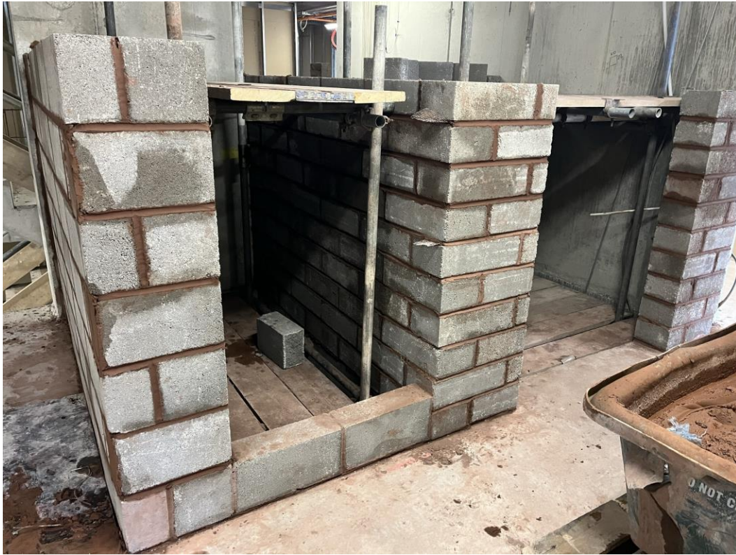
Lift shaft blockwork
