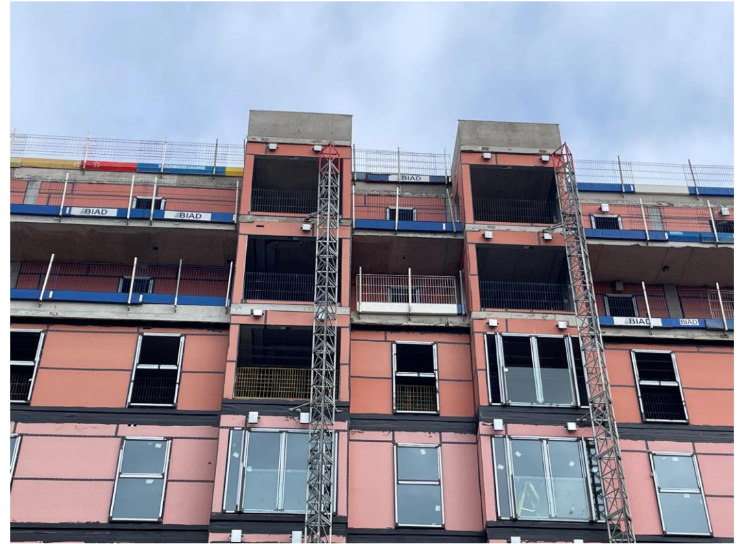
Block D Section B – External weatherboarding
