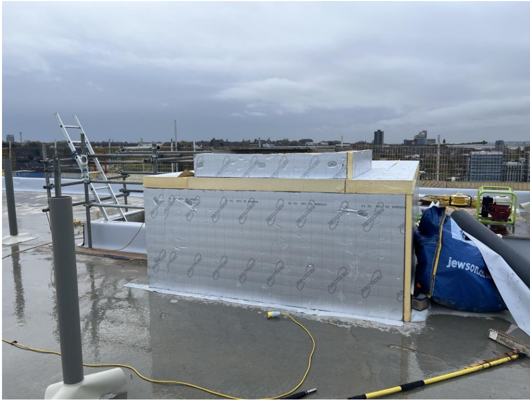
Block D Section B - Insulation boarding installed
