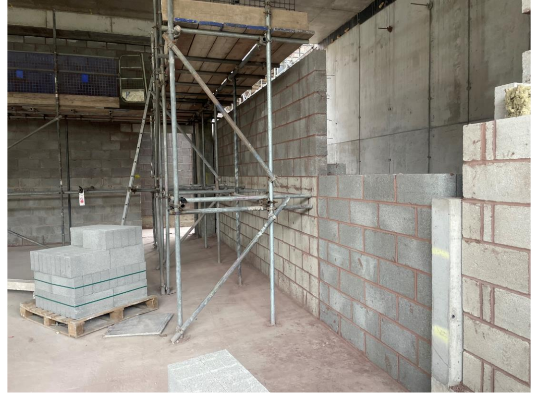
Ground floor blockwork wall
