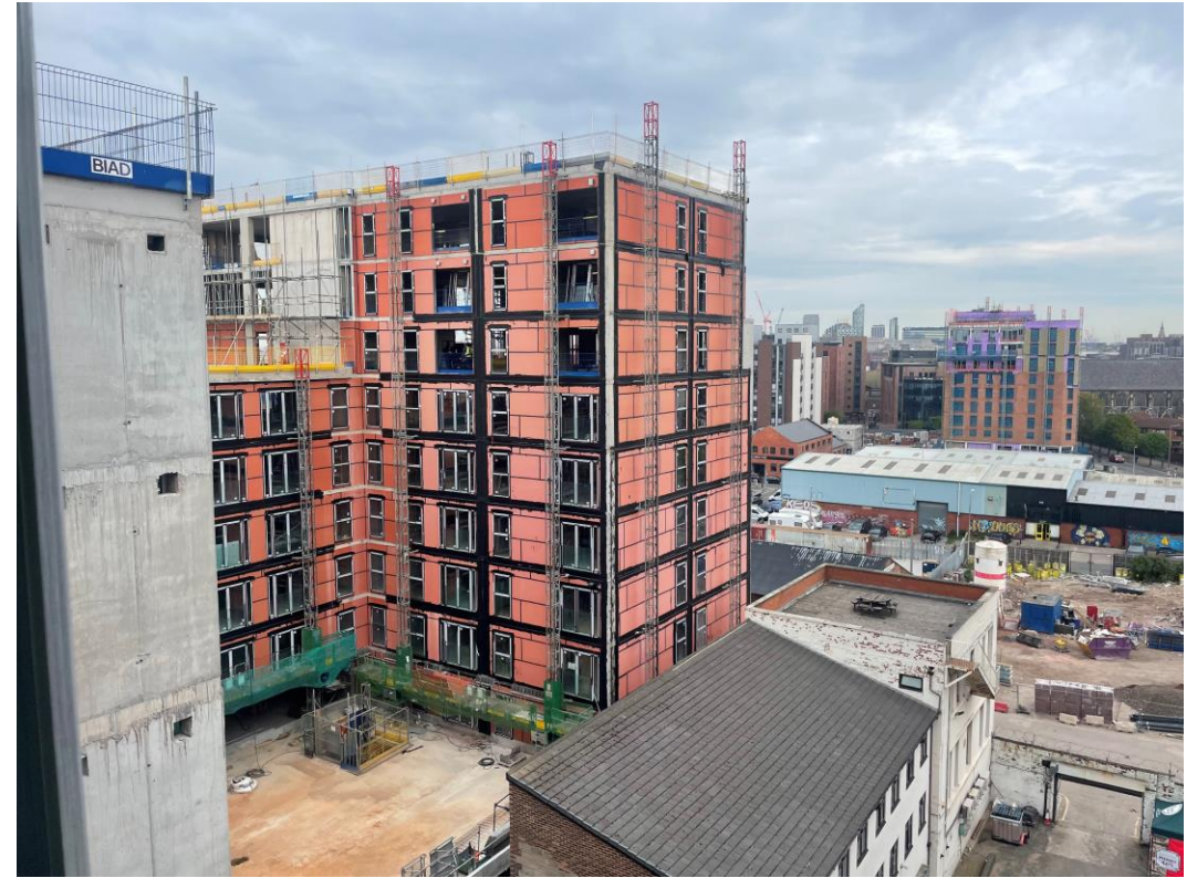
Block D Section B – SFS & Weatherboarding Installation
