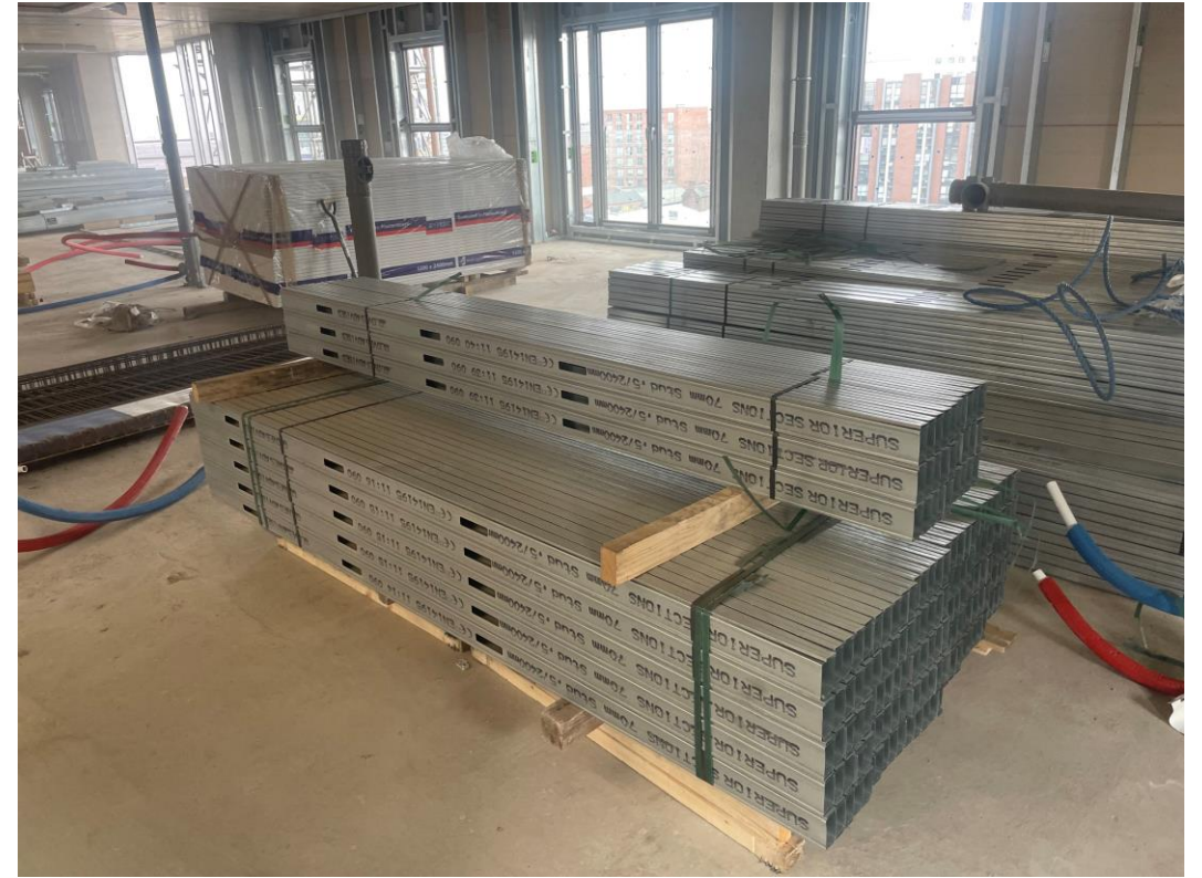
Metal partitions stored onsite for installation
