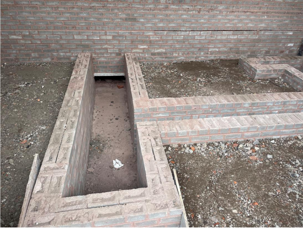
Ductwork channels formed to substation
