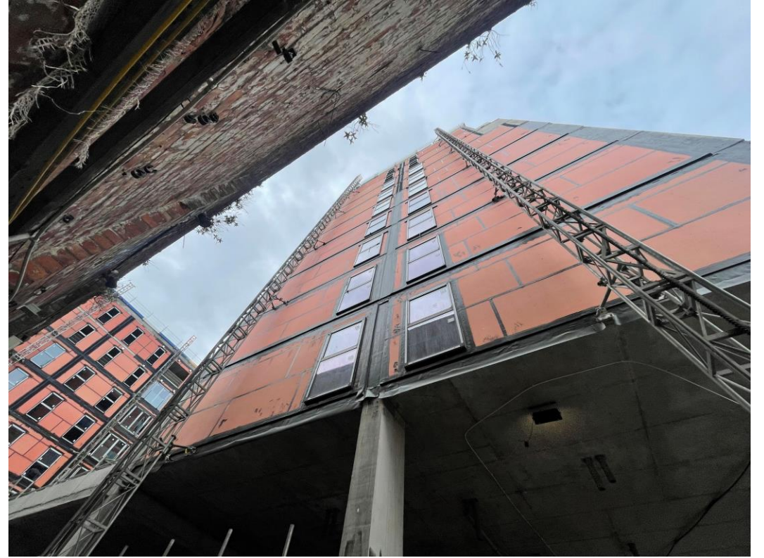
Block D Section B – Weatherboarding
