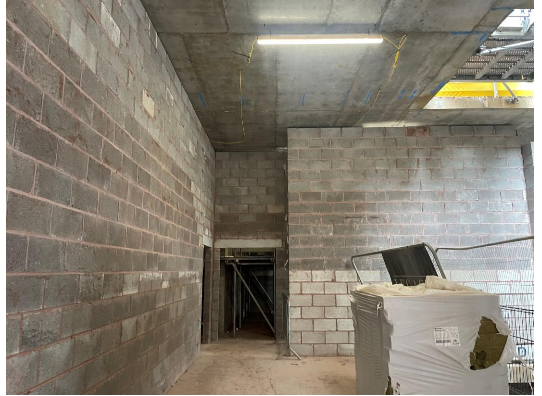
Ground floor blockwork wall
