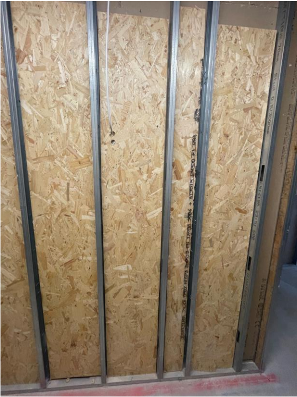
OSB board pattress installation commenced
