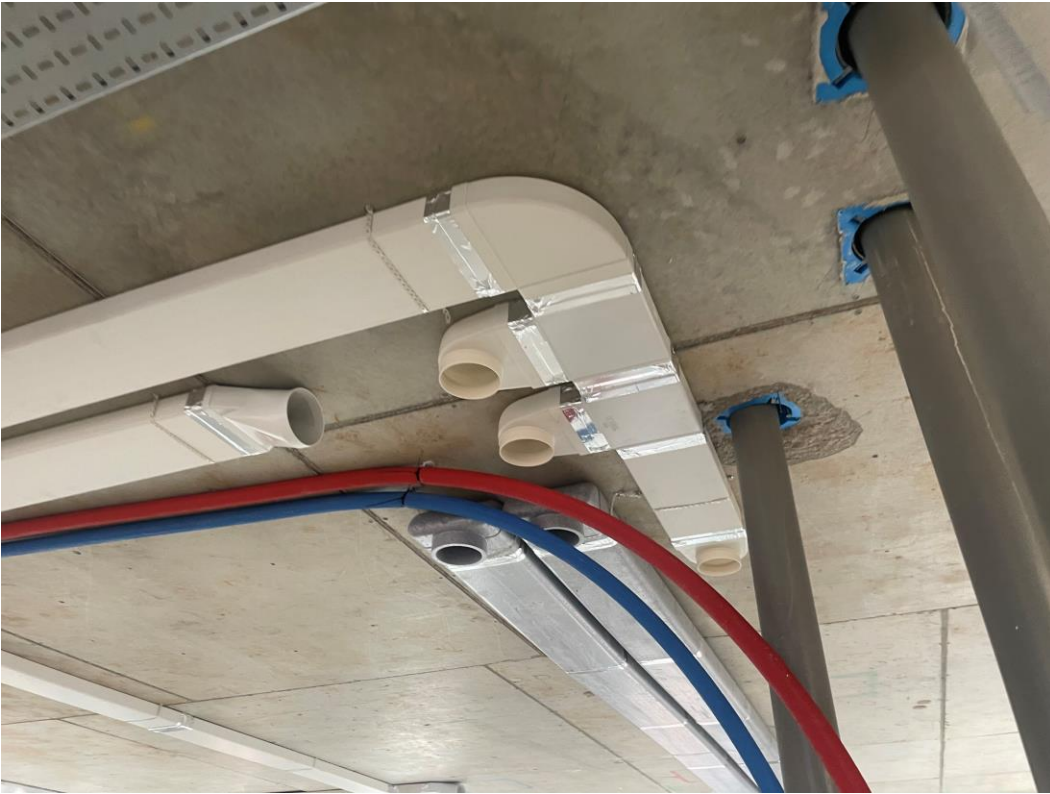
1 st Fix Mechanical ducting installation
