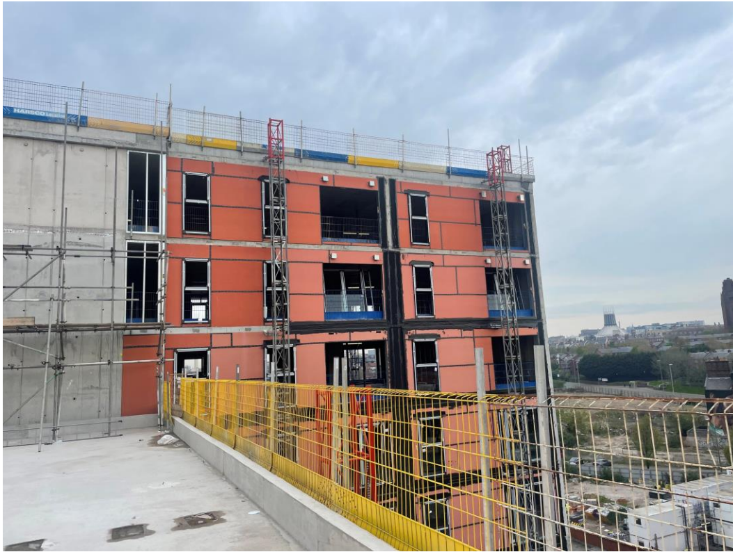
Block D Section A – SFS & Weatherboarding Installation
