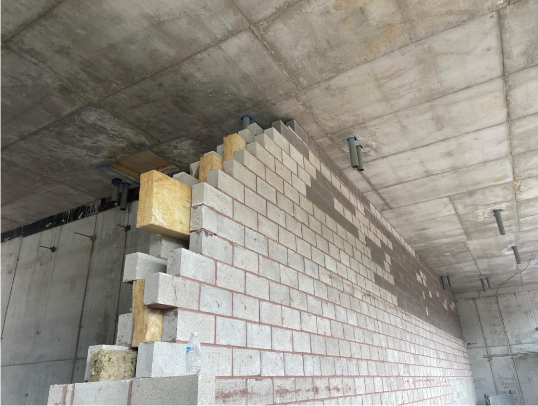
Ground floor blockwork wall
