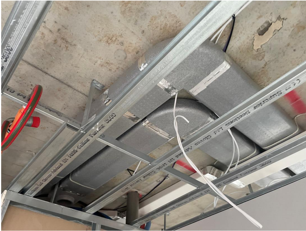
1 st Fix Mechanical ducting installation ongoing
