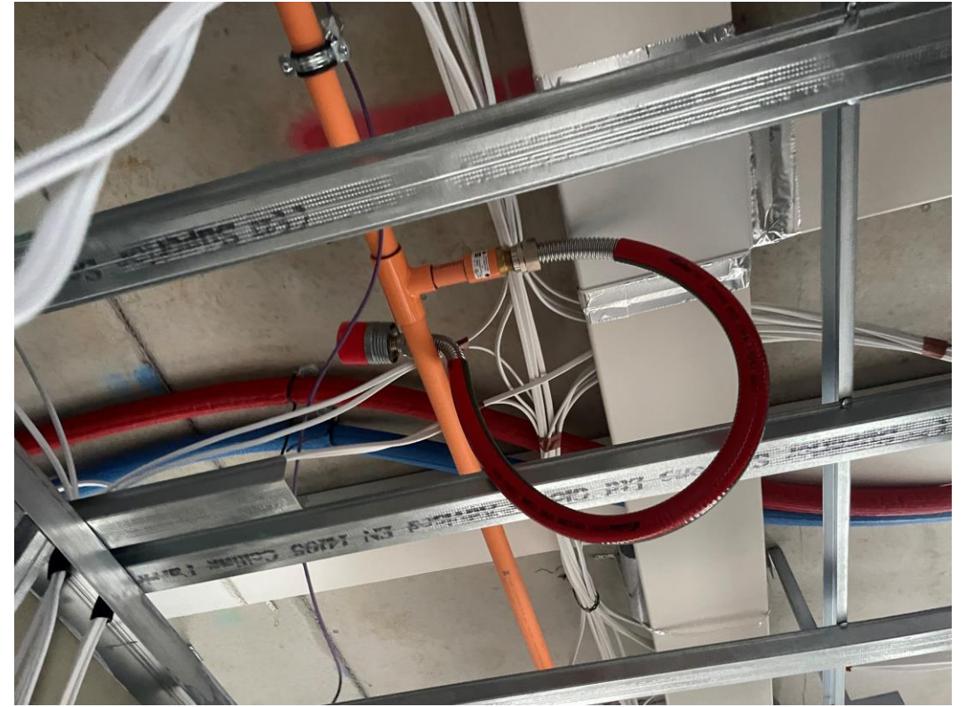
Sprinkler system installation ongoing
