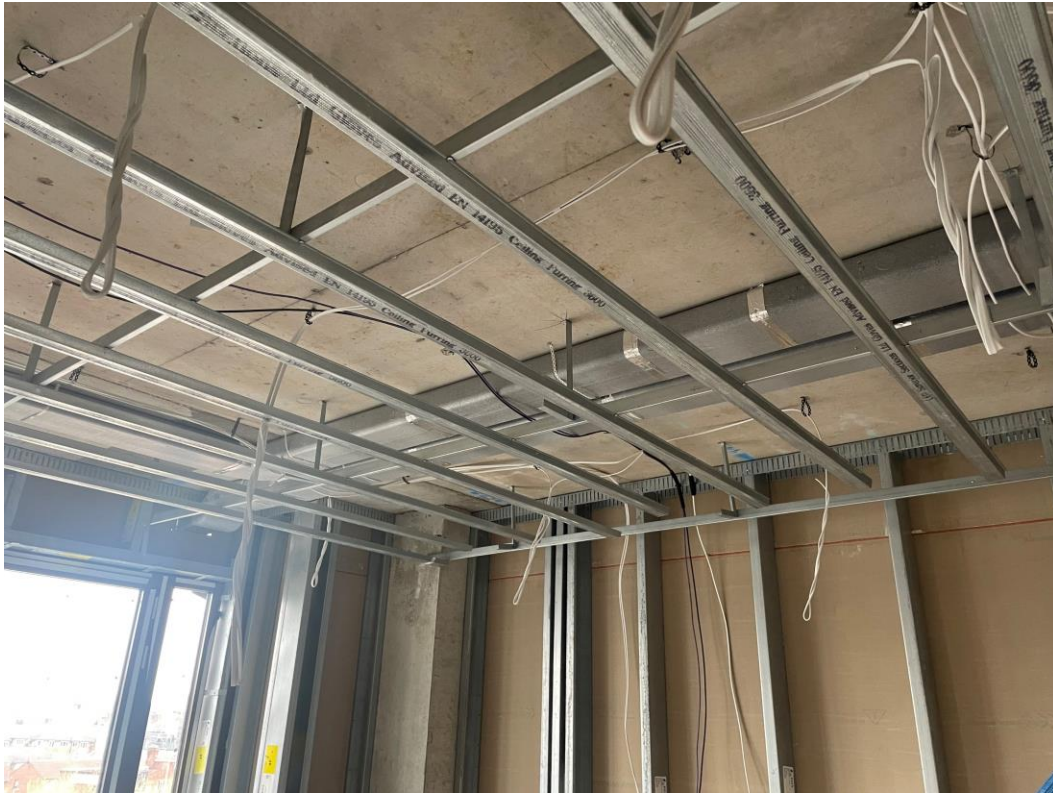
1 st Fix Electrical installation ongoing
