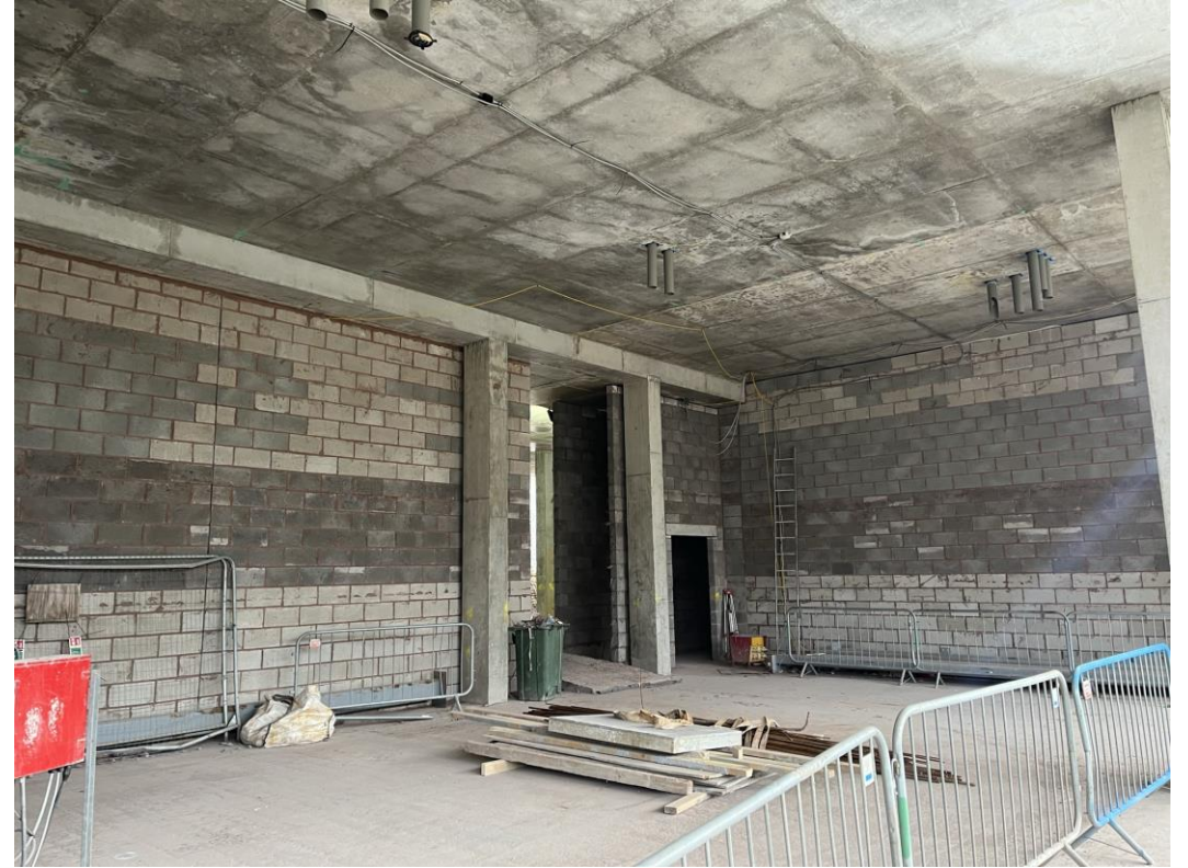
Blockwork walls formed
