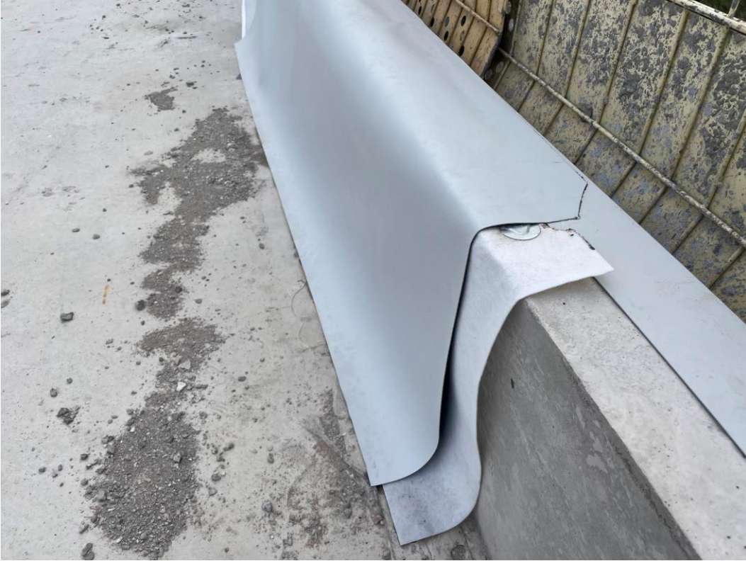
Block D Section B – Single ply membrane Installation
