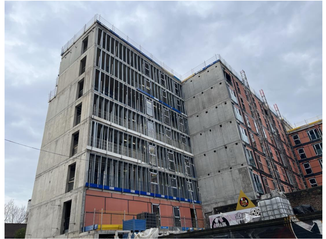
Block D Section B – SFS Installation
