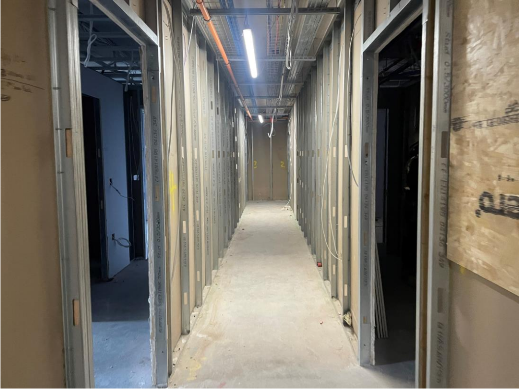
First side partition boarding ongoing
