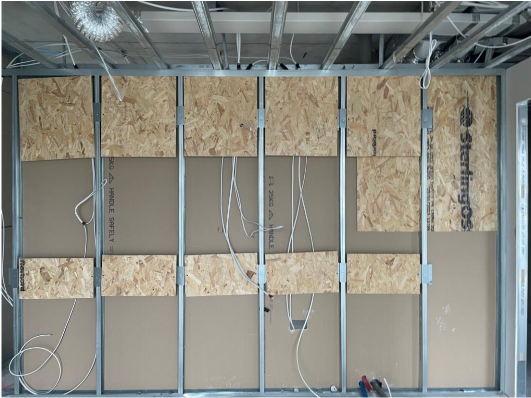
OSB board pattress installation commenced
