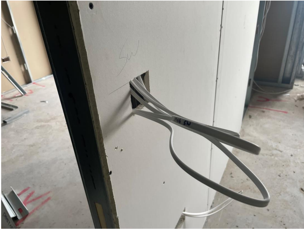
1 st Fix Electrical Installation
