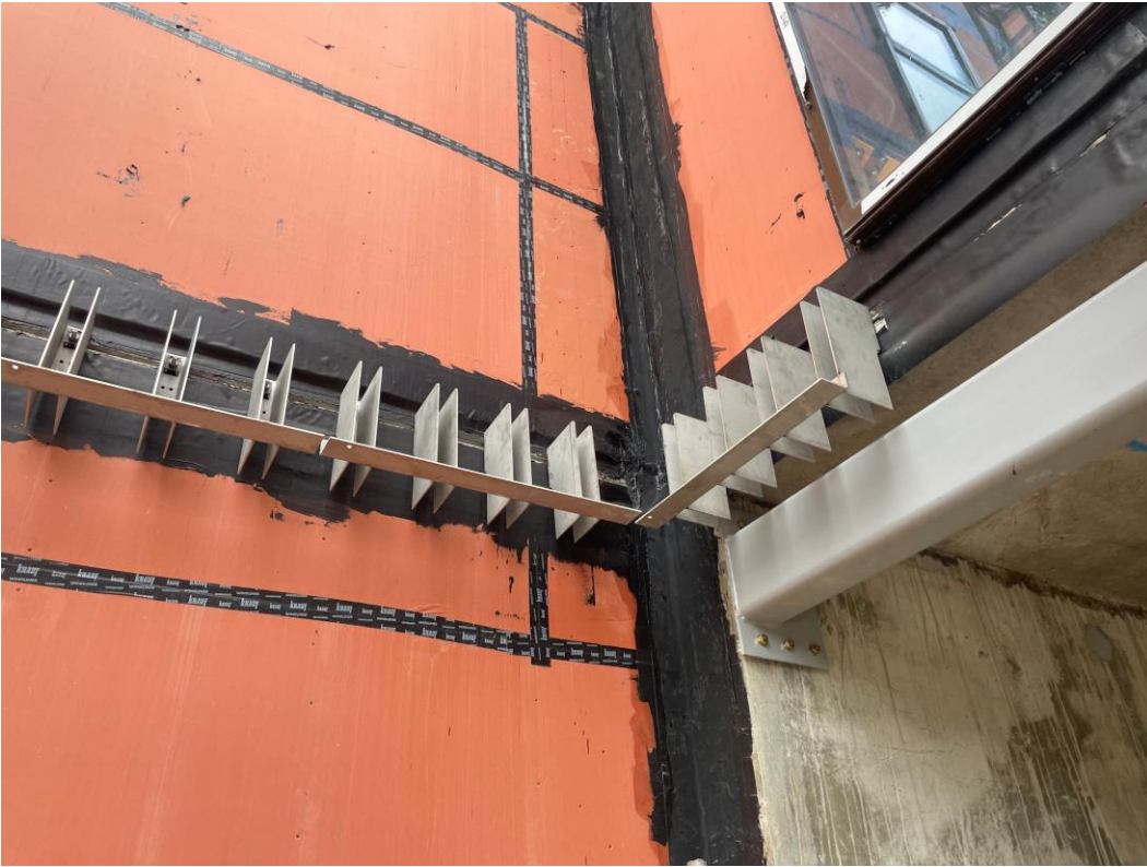
Block D – Masonry supports
