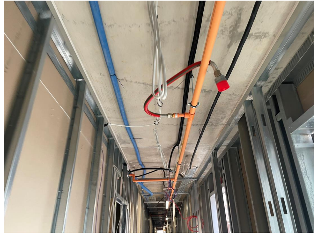
Sprinkler system installation ongoing
