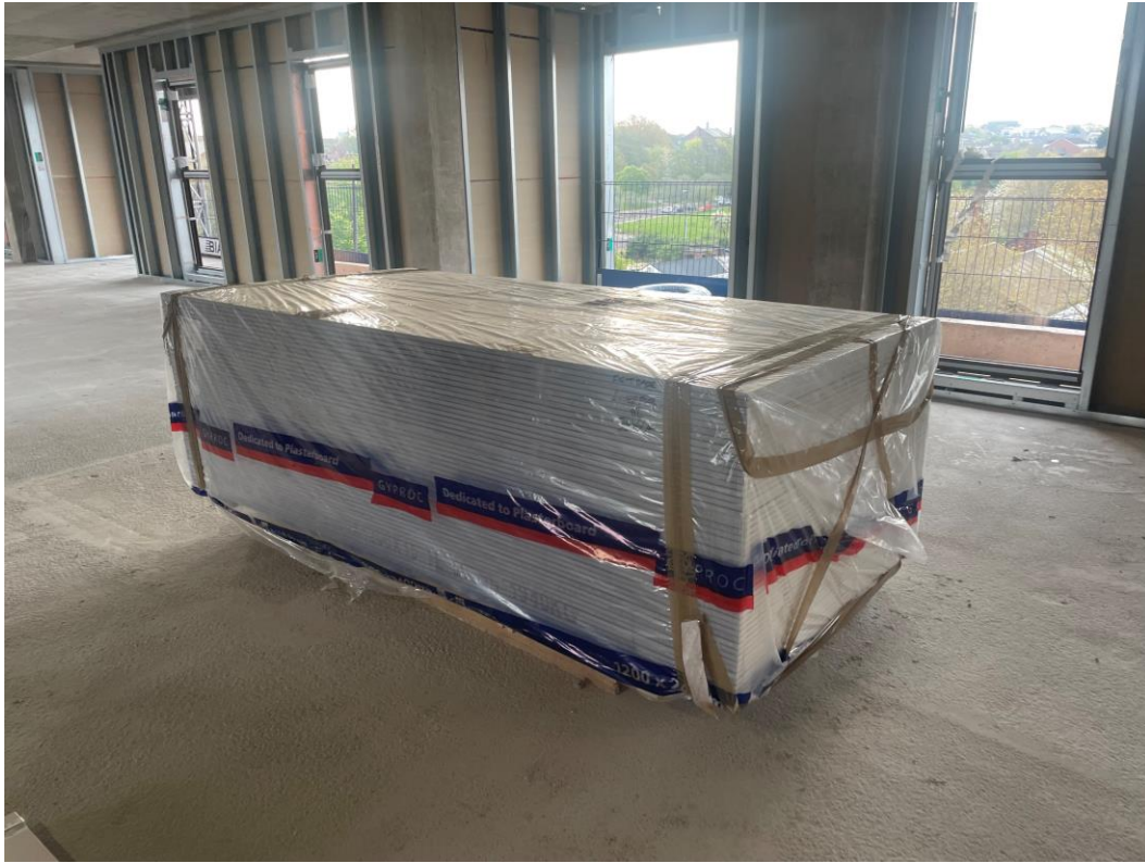
Plasterboard stored onsite for installation
