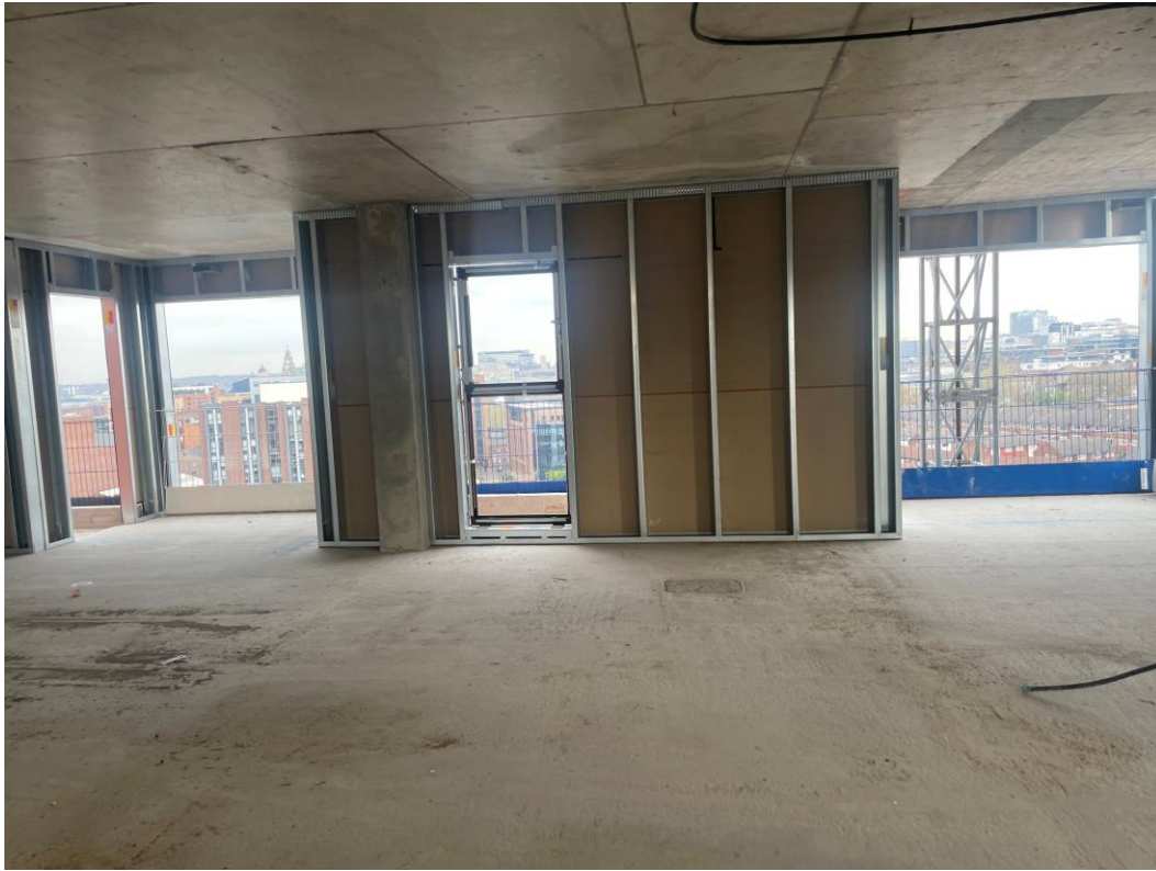
SFS installation nearing completion
