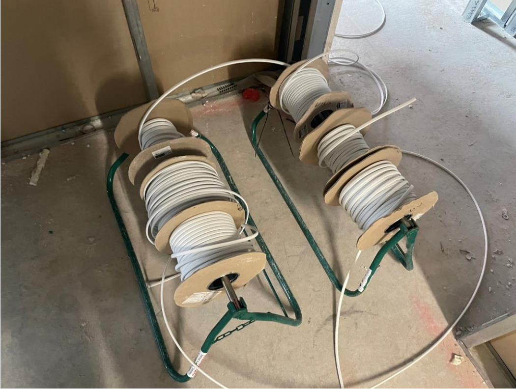
1 st Fix electrical cabling
