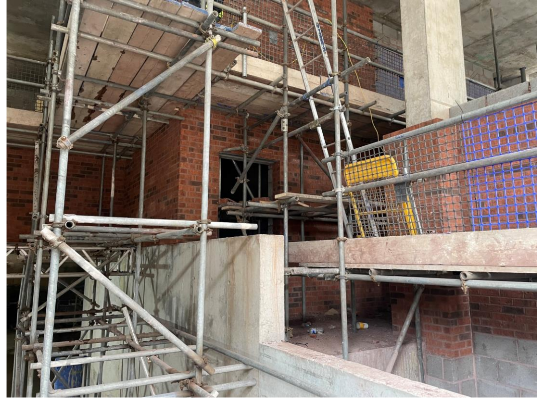
Ground floor brickwork walls
