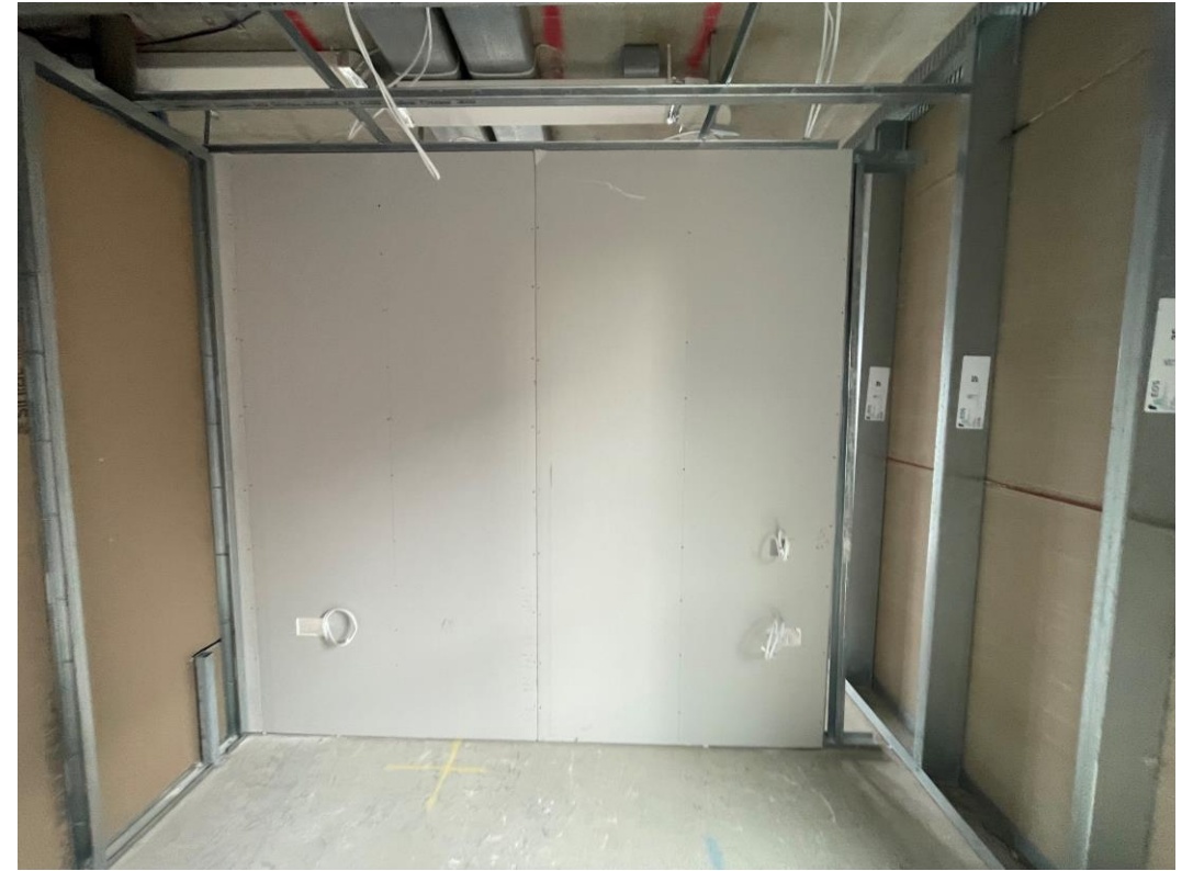
First side partition boarding ongoing
