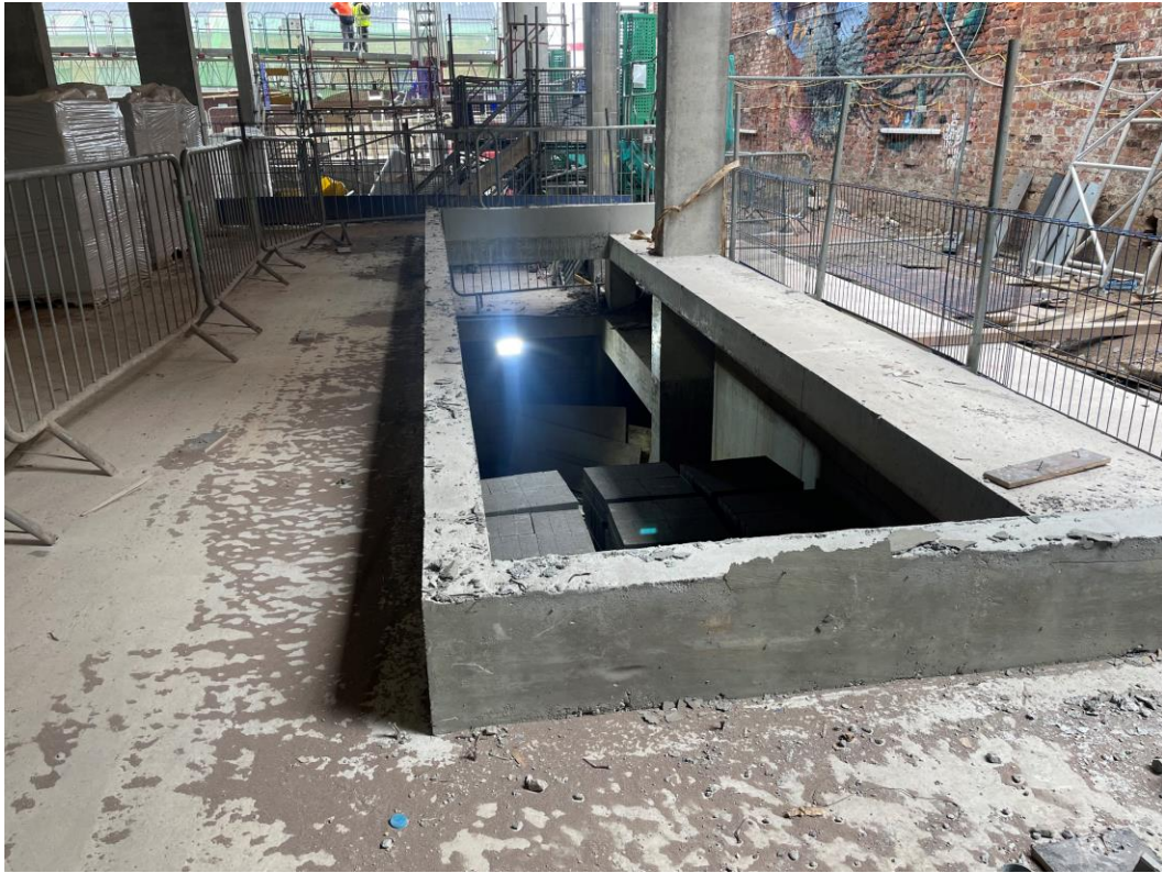
Concrete upstand in place
