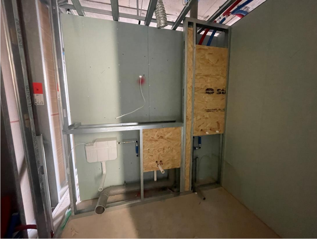
Metal IPS installation ongoing
