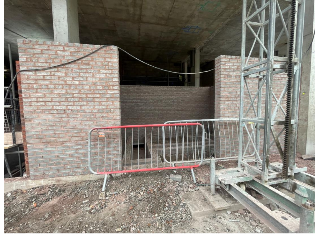
Substation substructure brickwork
