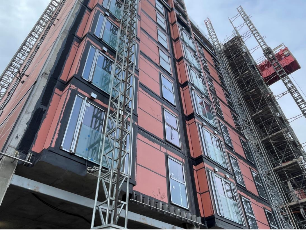
Block D Section A – Window units
