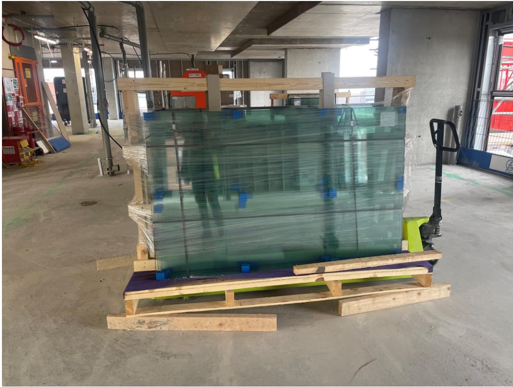
Glazing units on site for installation
