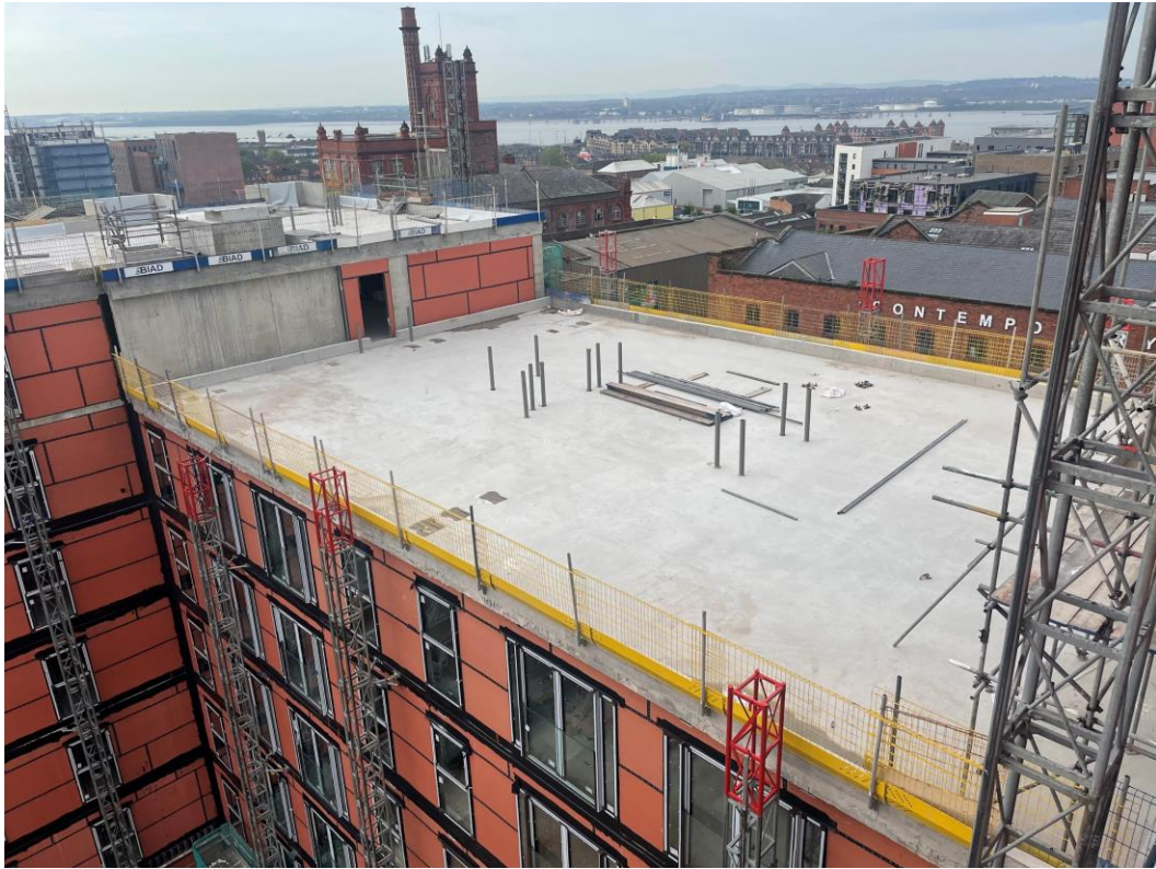
Block D Section C – Roof
