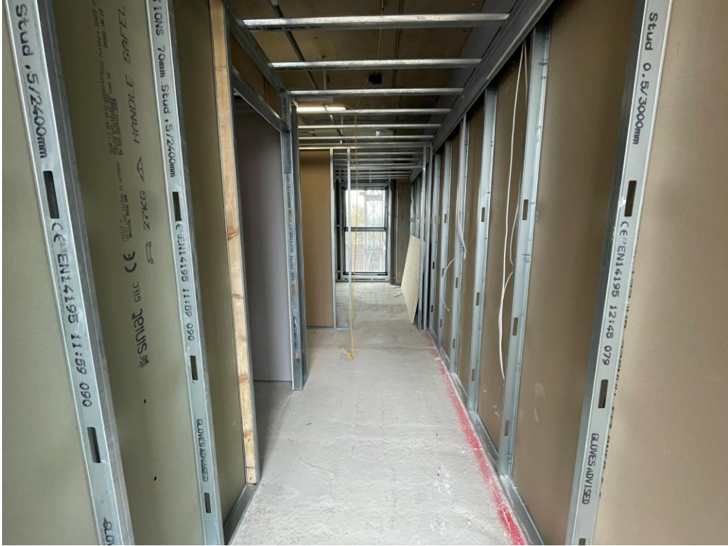
First side partition boarding ongoing
