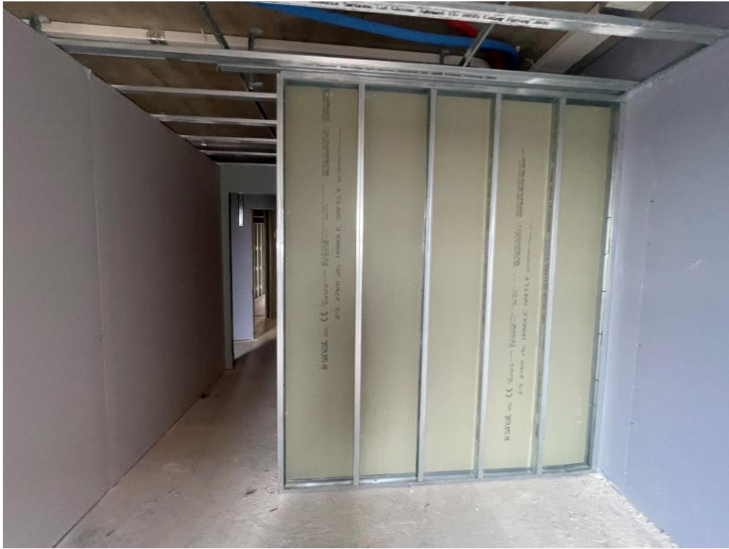
First side partition boarding ongoing
