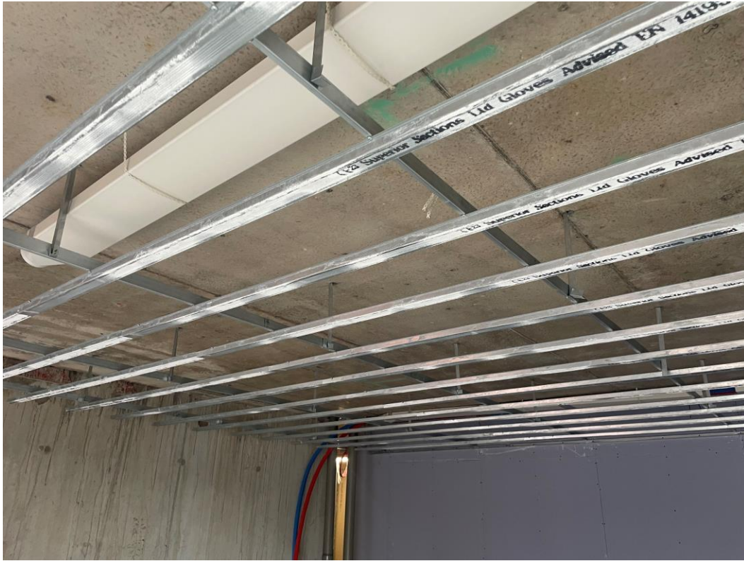
Ceiling grid installation ongoing
