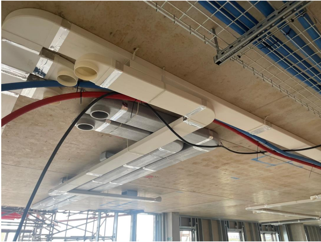
1 st Fix Mechanical ducting installation ongoing
