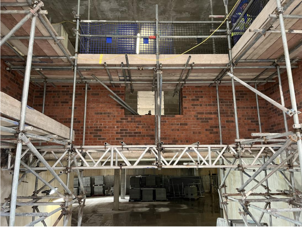
Ground floor brickwork walls
