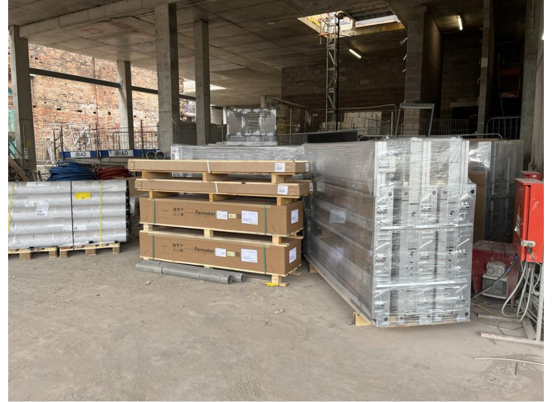
Lift components stored onsite for installation
