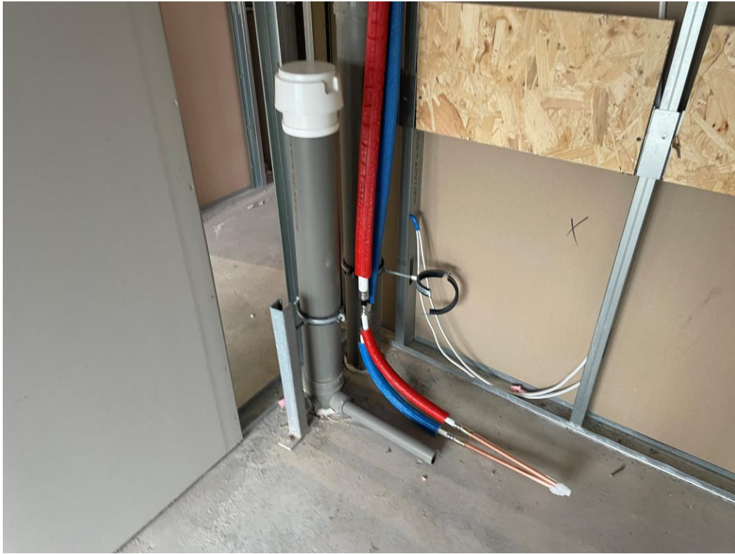
Apartment hot & cold water feed installation ongoing
