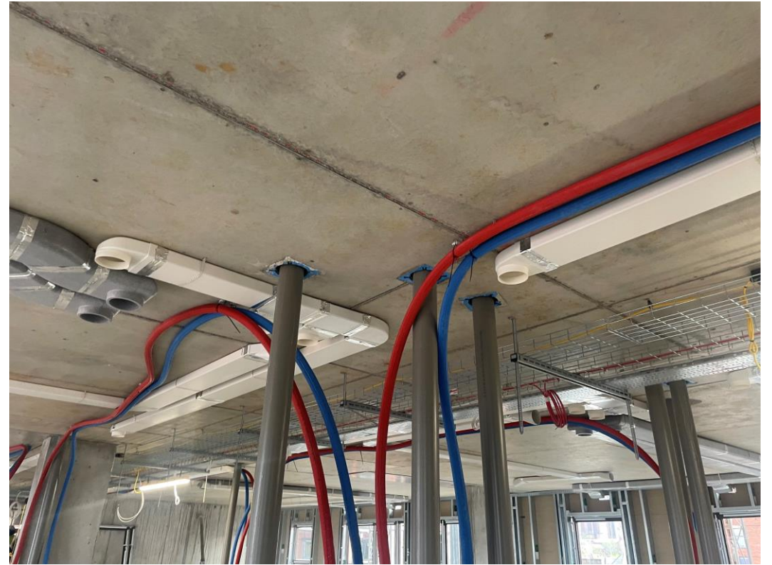
1 st Fix Mechanical ducting installation
