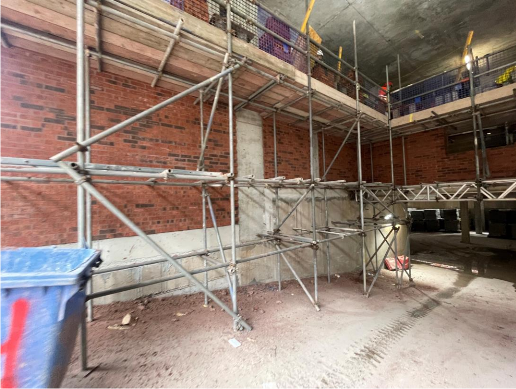
Ground floor blockwork walls
