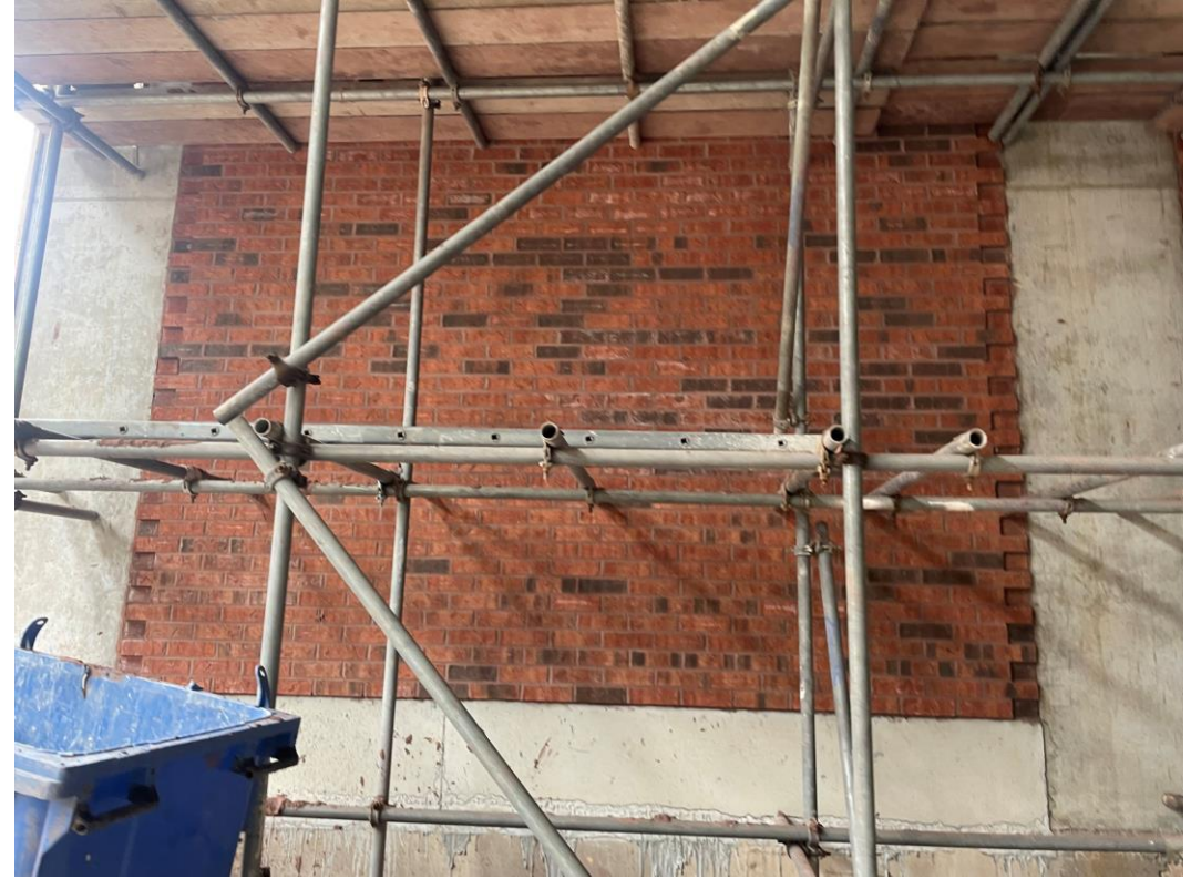
Ground floor brickwork walls
