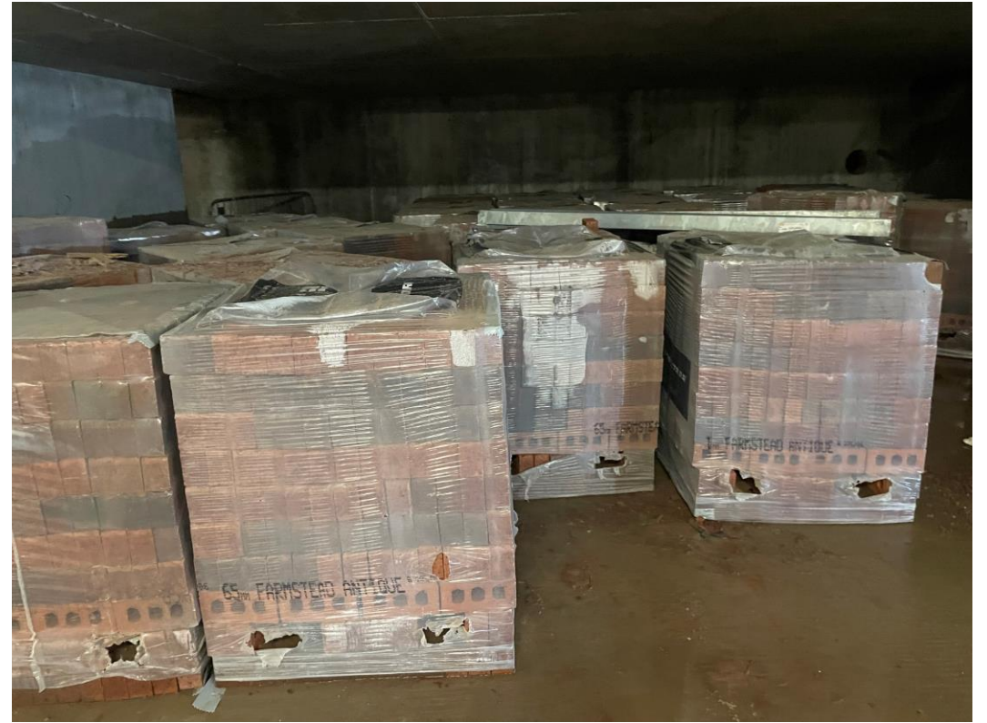
Bricks stored onsite for installation
