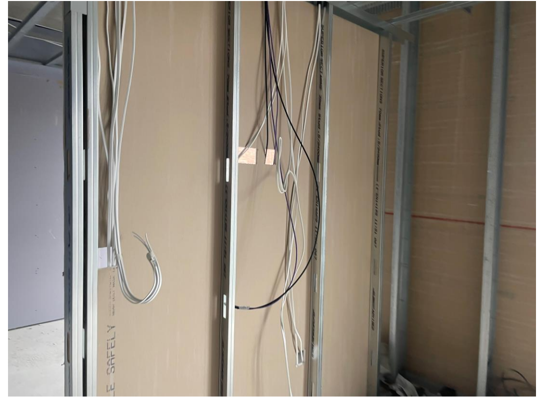
1 st Fix Electrical installation ongoing
