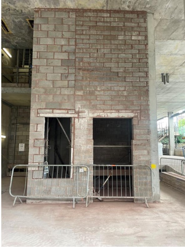
Ground floor blockwork lift shaft
