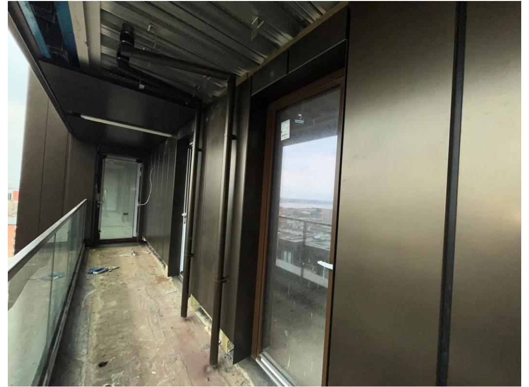
Rain water pipes & cladding installation ongoing
