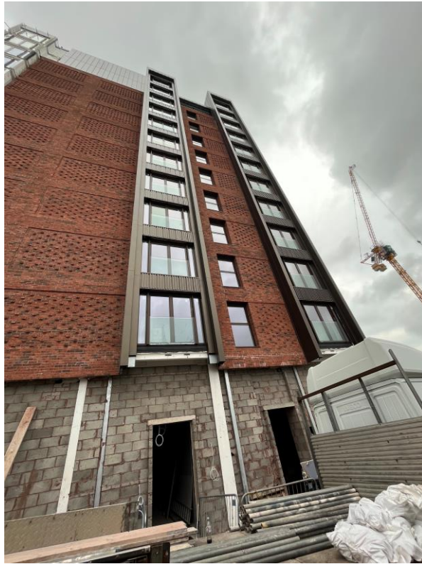
Block B – Brickwork & cladding installation
