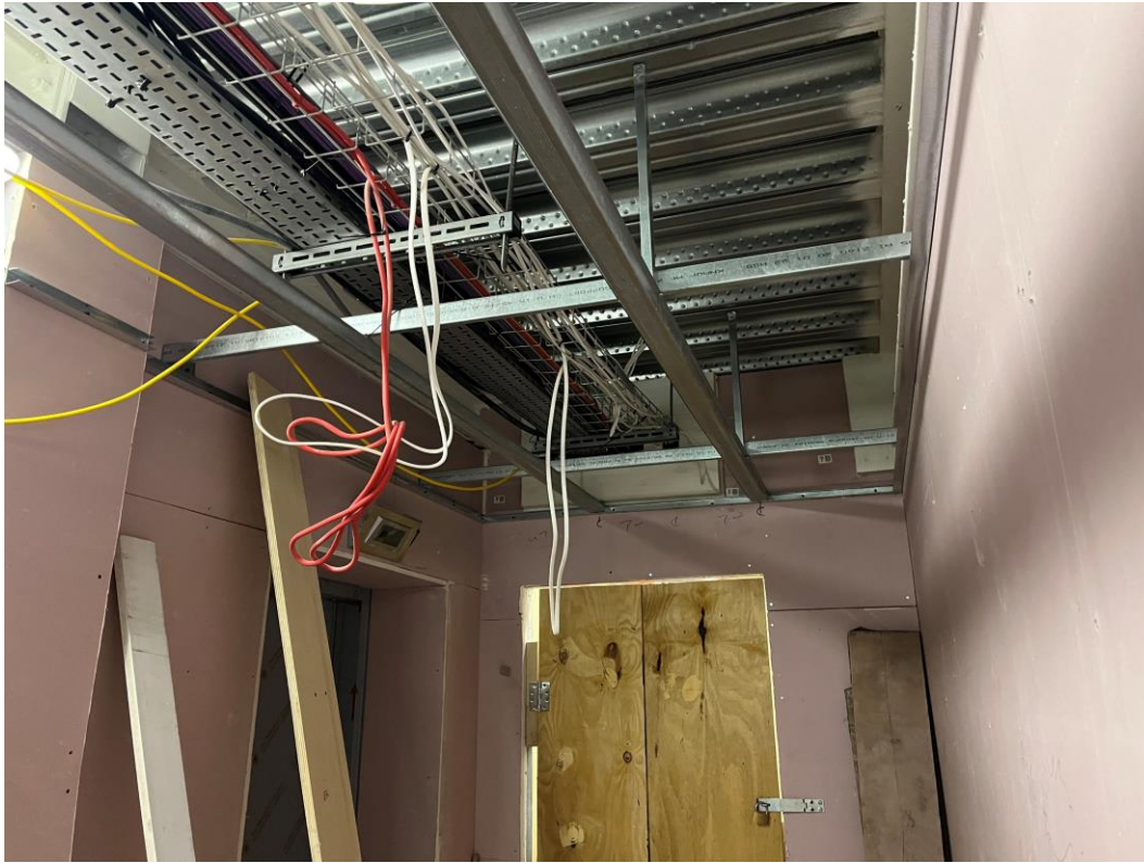
Ceiling grid erected to circulation areas
