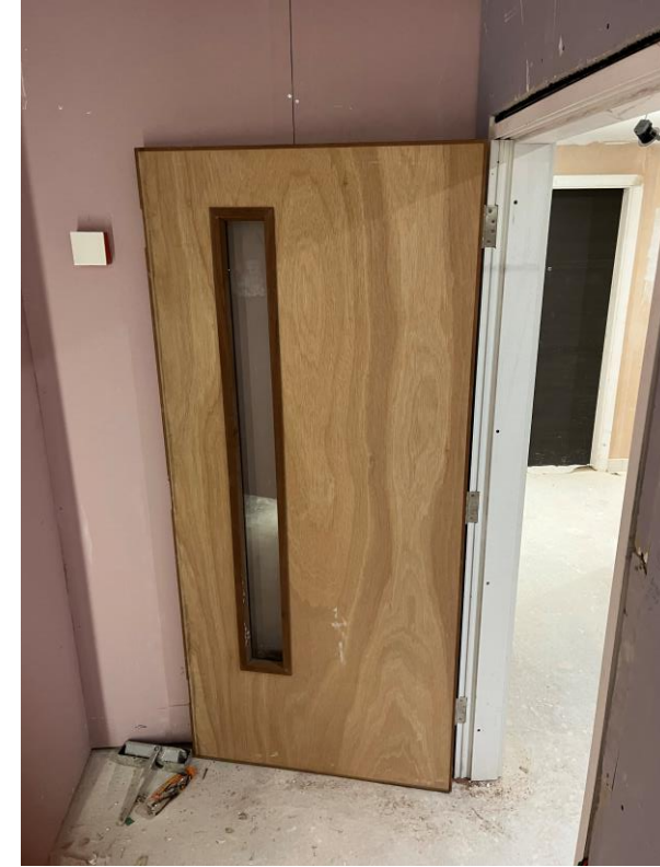
Fire doors installed
