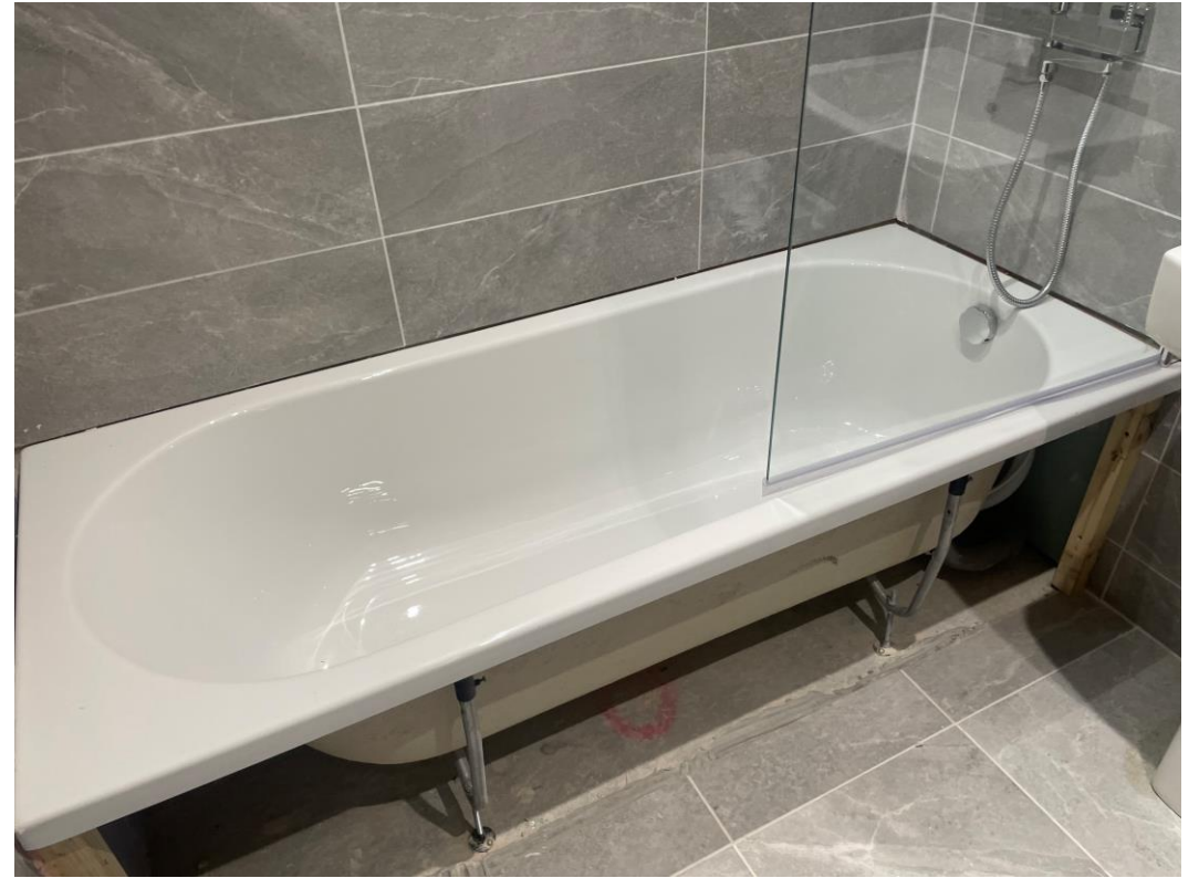
Bathroom appliances installed
