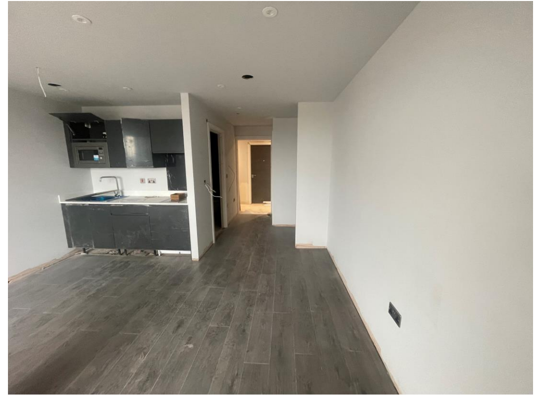
Kitchen / Lounge finishes
