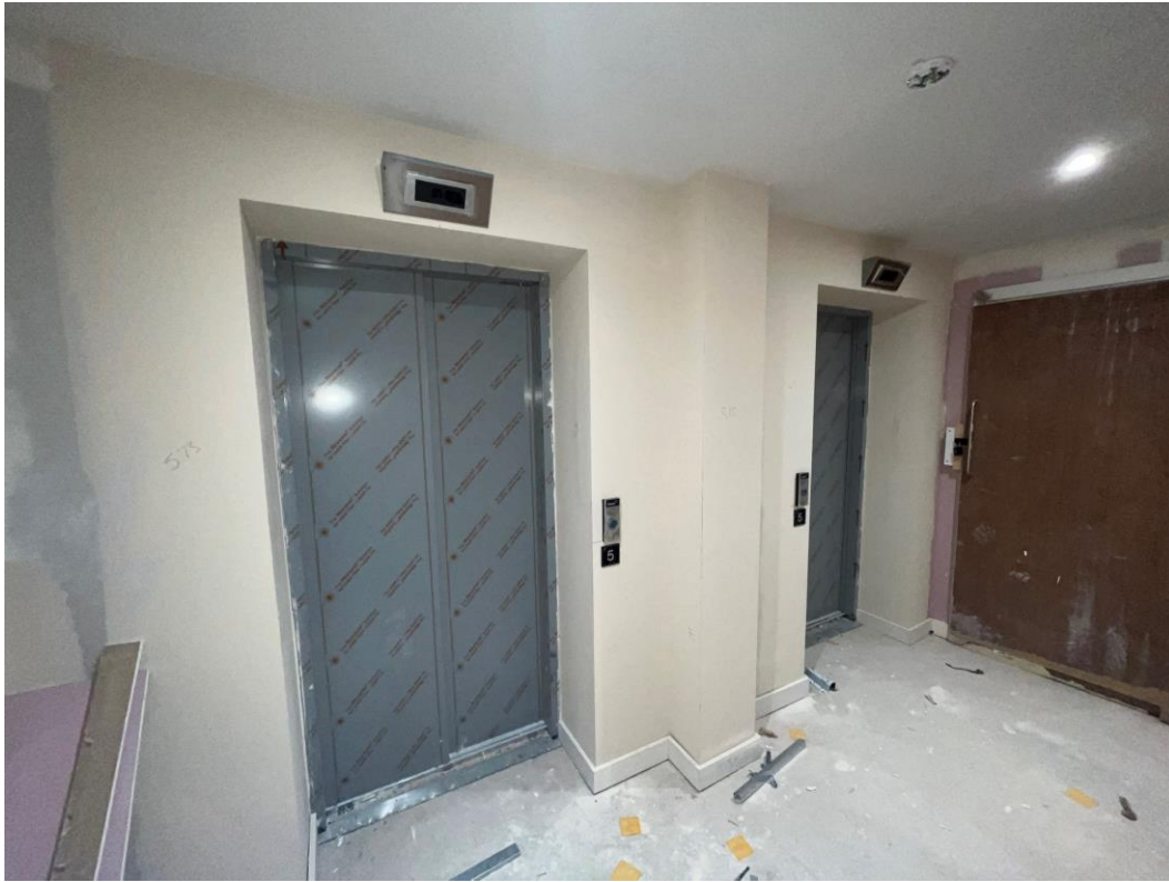
Walls & ceilings plastered to lift area
