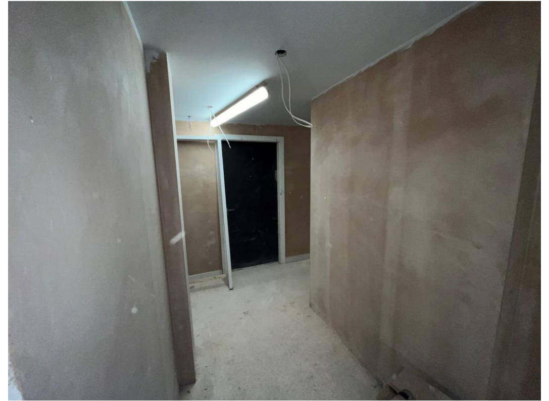
1 st coat decoration to ceilings
