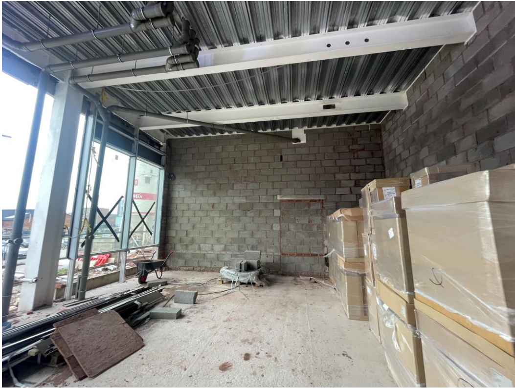
Masonry wall installed to Commercial Unit
