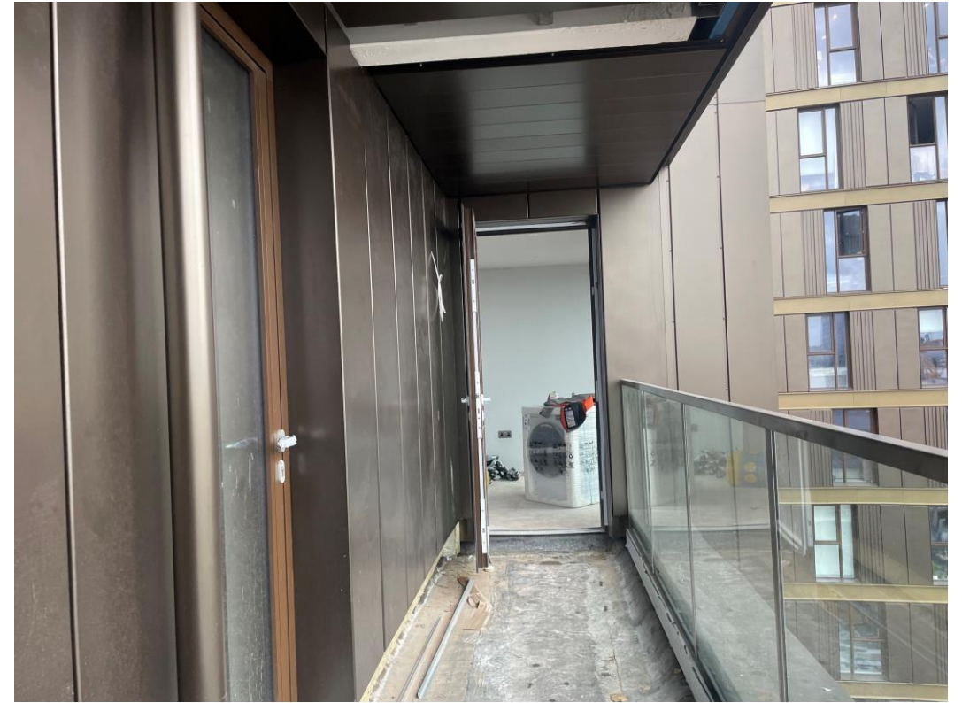
Cladding installation ongoing
