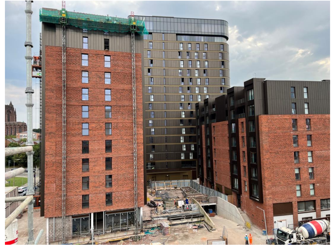
Block B – Viewed from Block D
