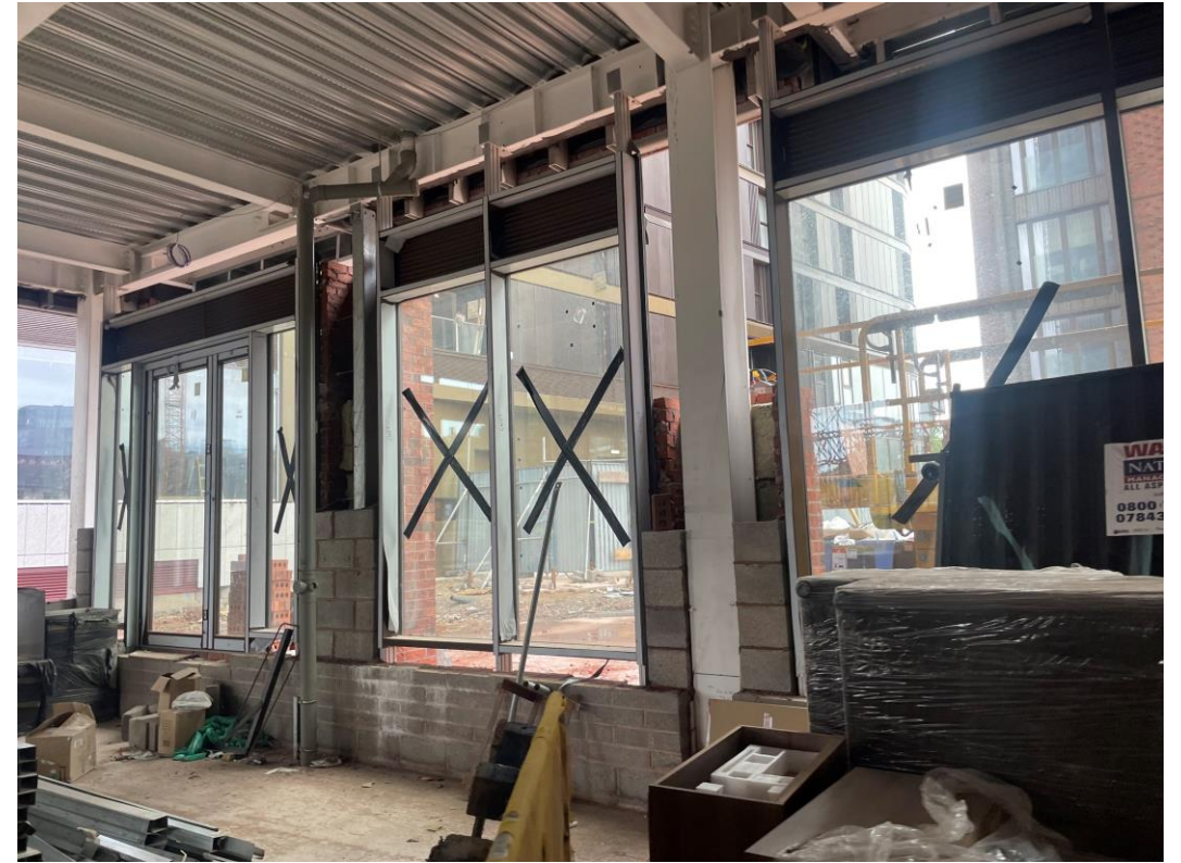
Curtain walling installed
