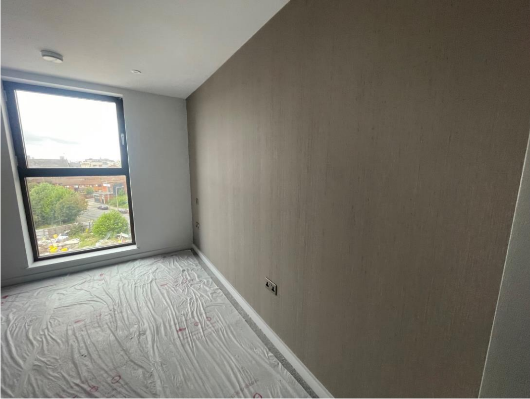
Bedroom feature wall installed
