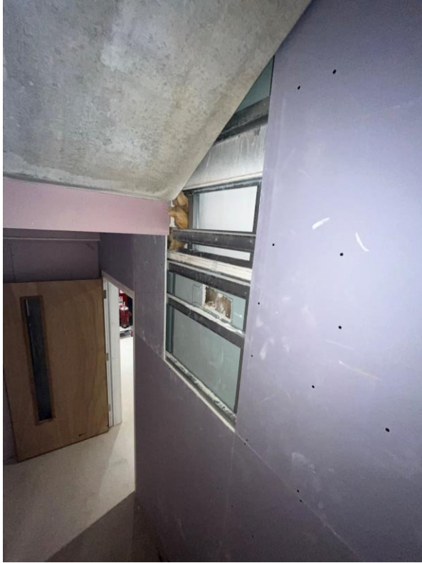
Boarding ongoing to stairwell
