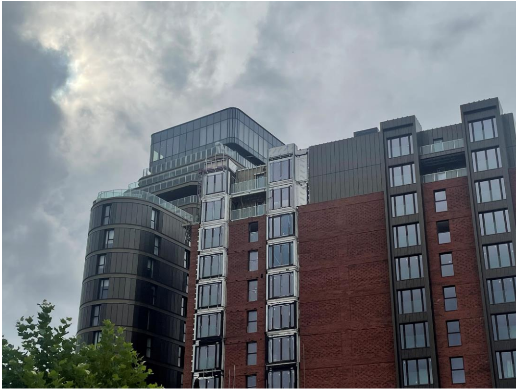
Block B – Brickwork & cladding installation
