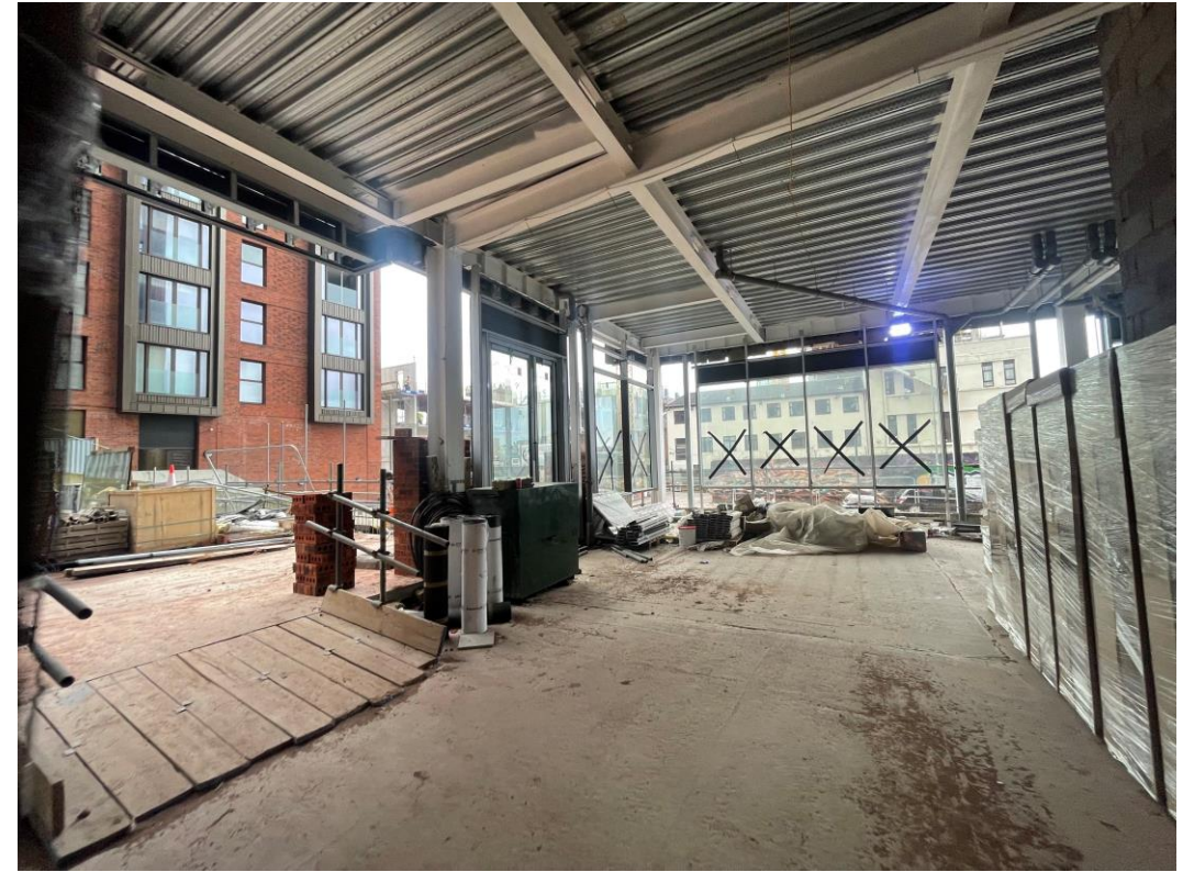
Curtain walling installed
