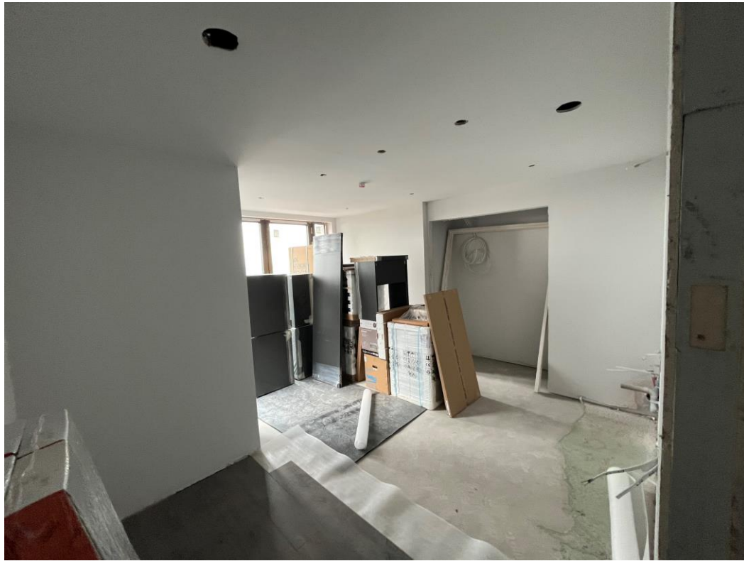
Lounge finishes ongoing
