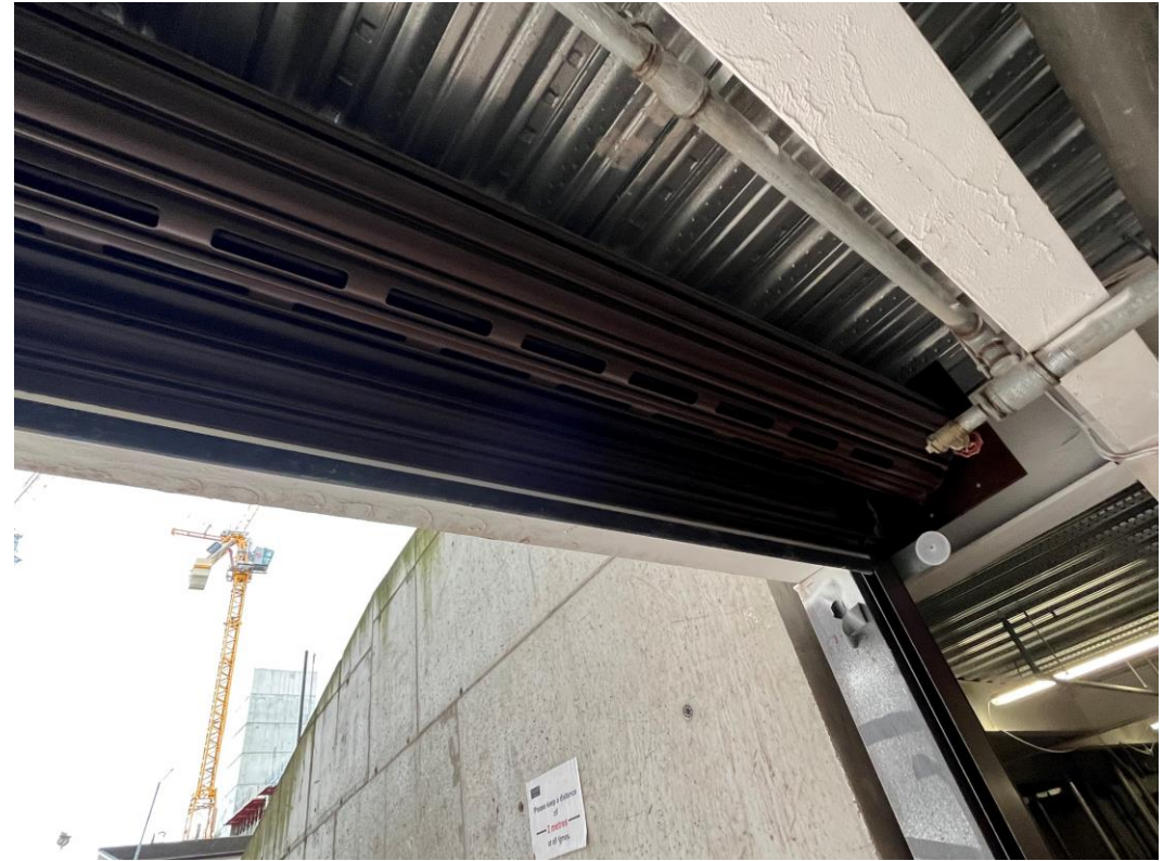
Roller shutter installed
