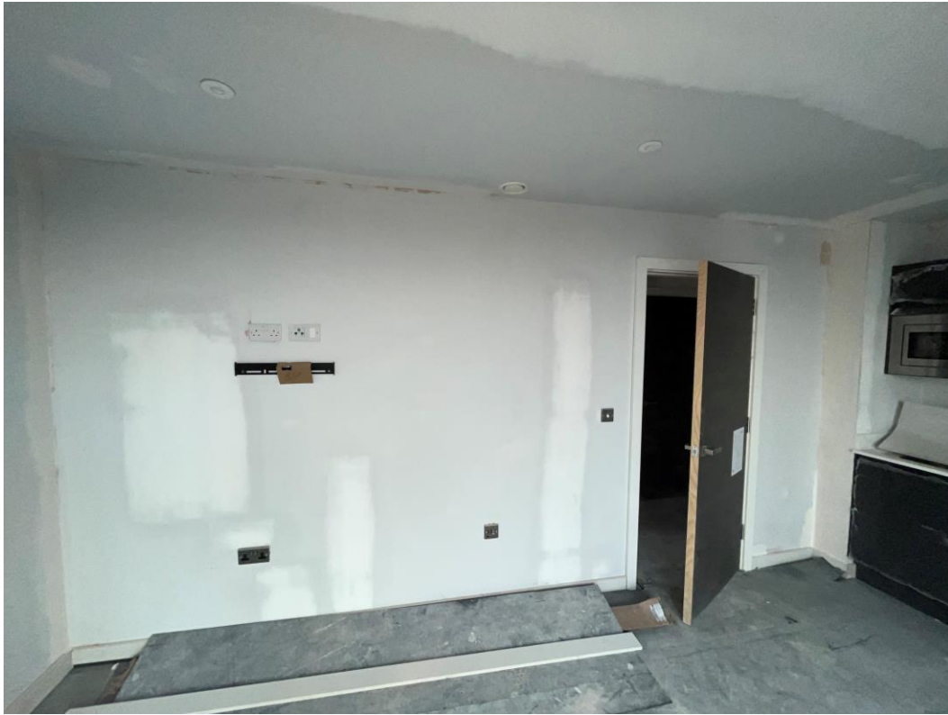
1 st coat decoration to wall & ceiling
