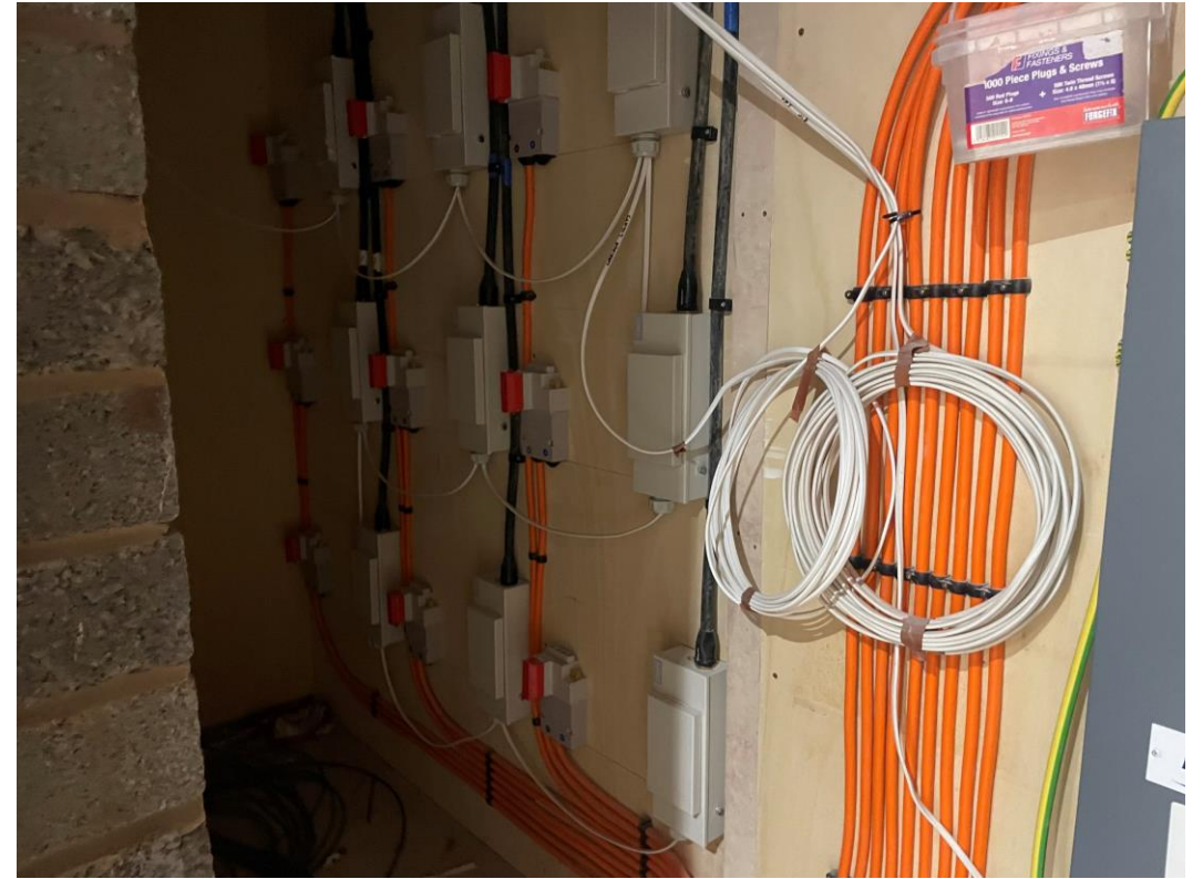
Electrical meters installed
