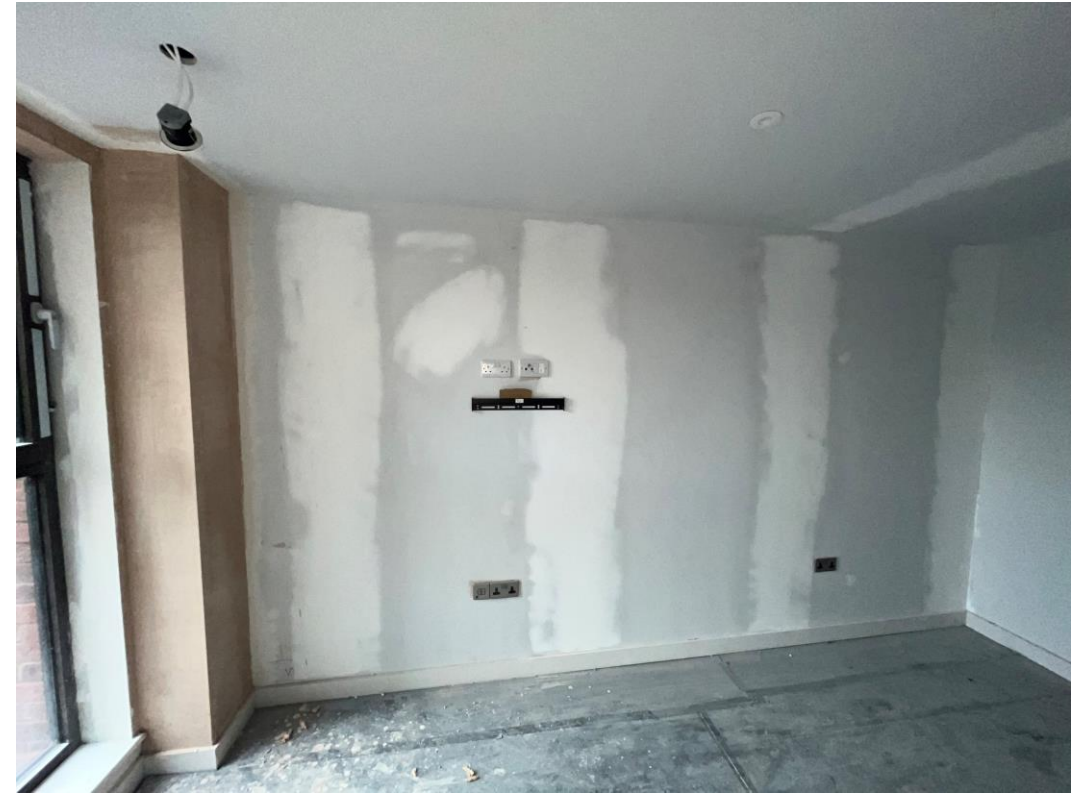
1 st coat decoration to walls & ceilings
