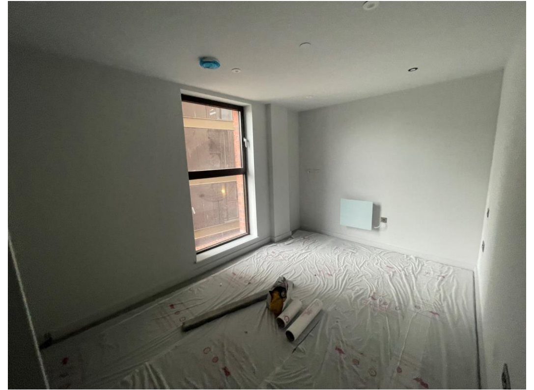
2 nd Coat decoration walls & ceilings
