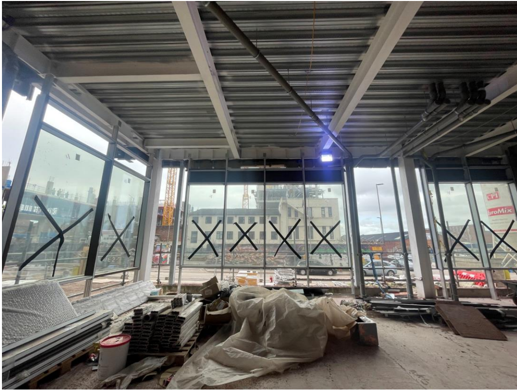
Curtain walling installed
