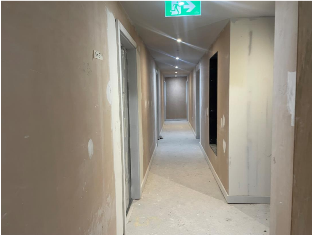
Circulation areas plastered
