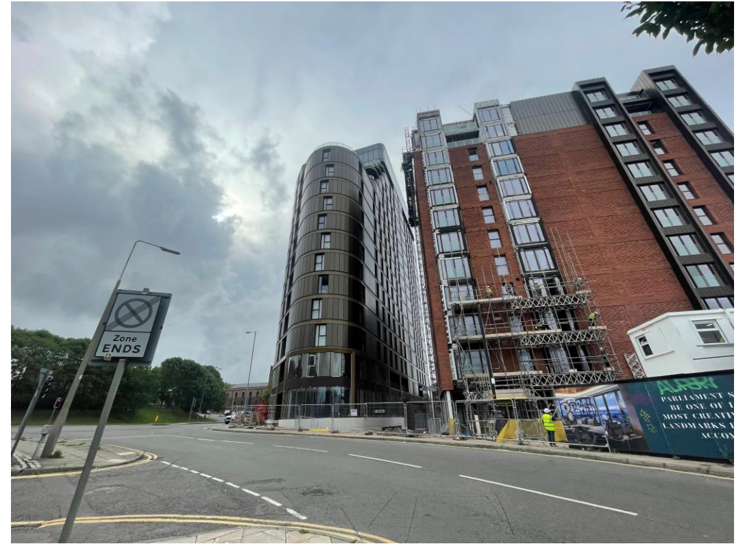
Block B – Brickwork & cladding installation
