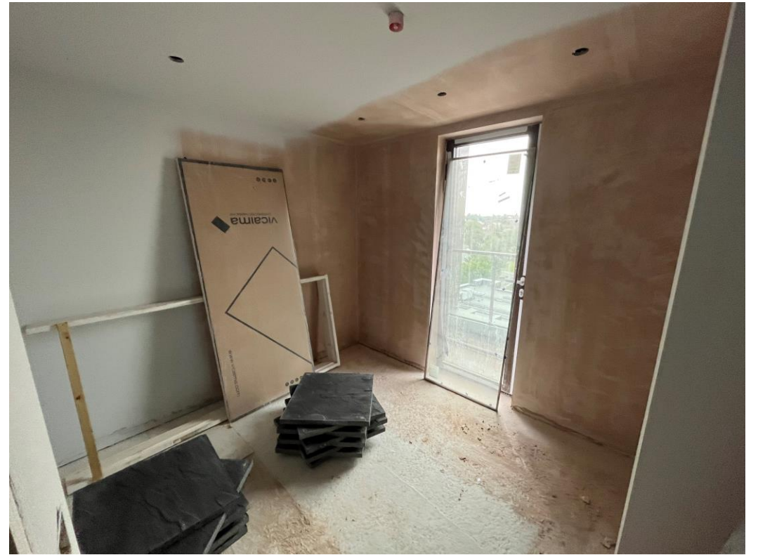
1 st coat decoration to wall & ceiling
