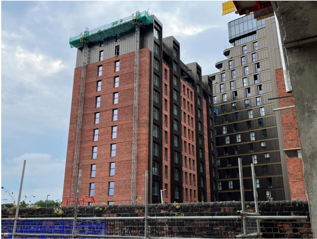
Block B – Viewed from Block D
