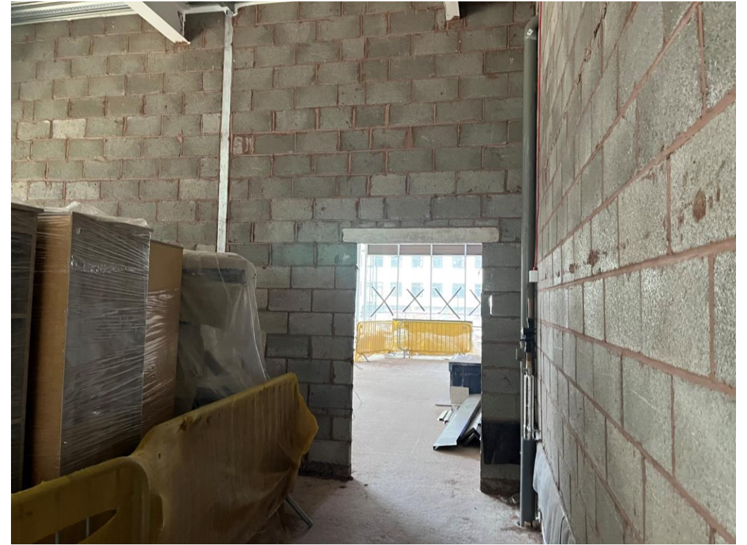
Masonry wall installed to Commercial Unit
