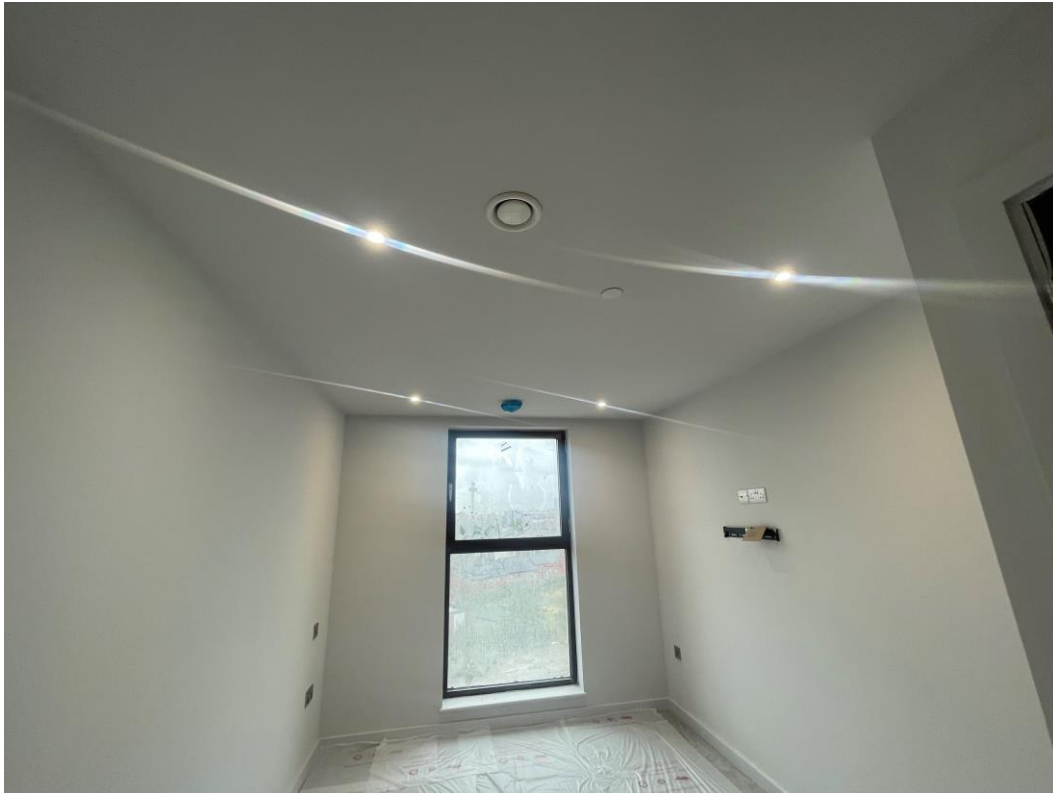
2 nd Coat decoration walls & ceilings
