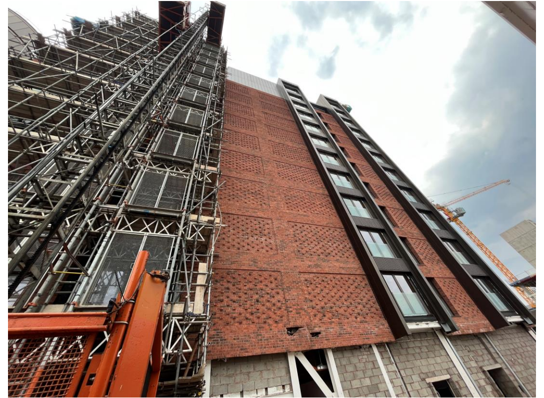
Block B – Brickwork & cladding installation
