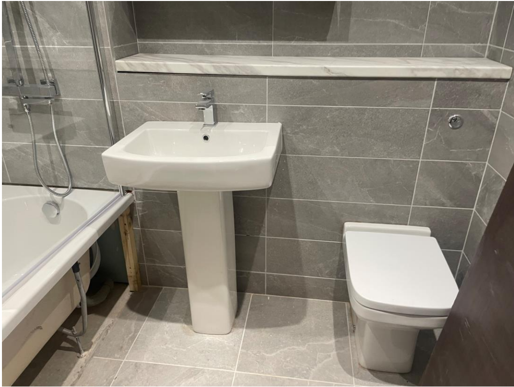
Bathroom appliances installed
