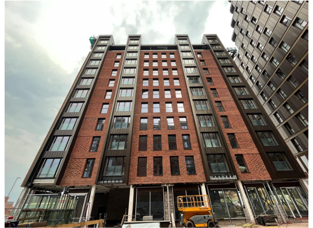
Block B – Brickwork & cladding installation
