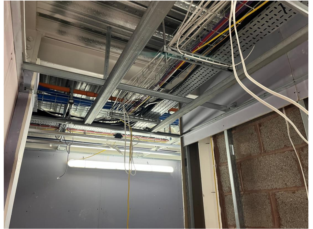
Ceiling grid erected to circulation areas
