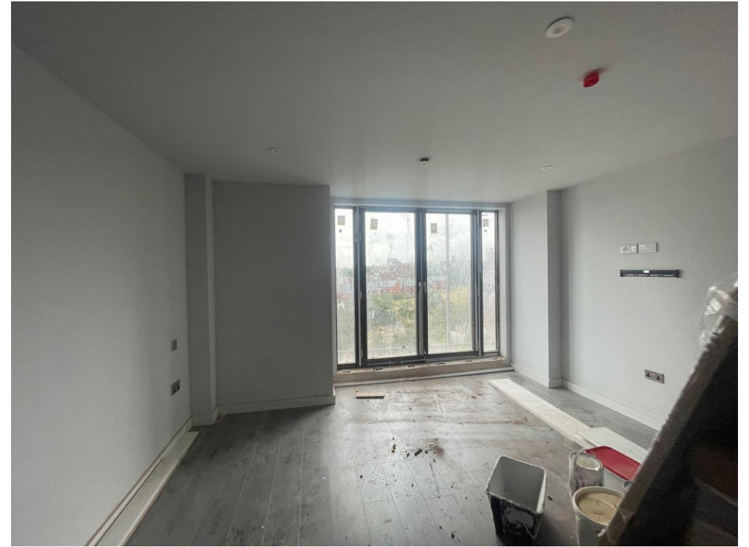
Lounge finishes ongoing
