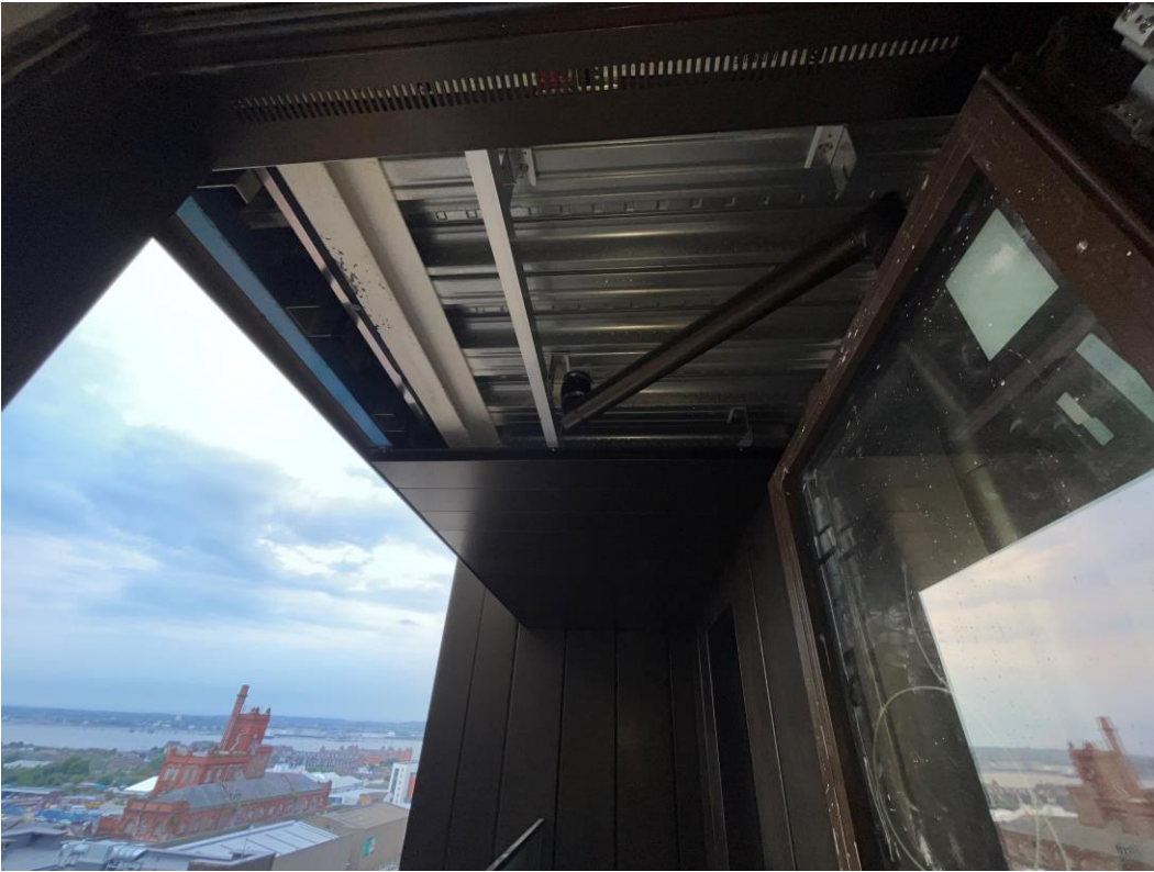
Soffit cladding installation ongoing
