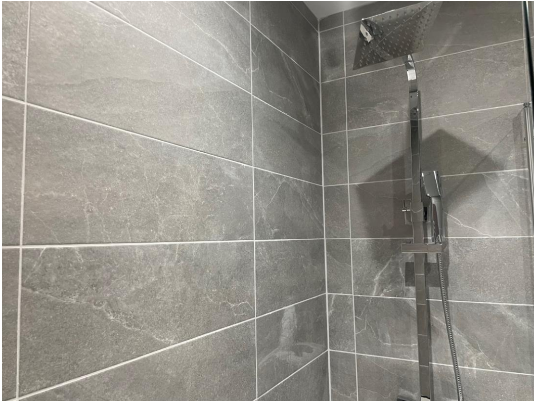
Bathroom appliances installed
