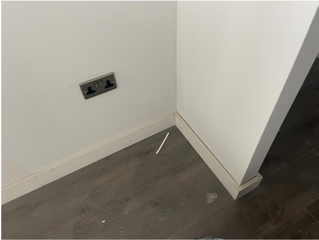
Skirting board installed
