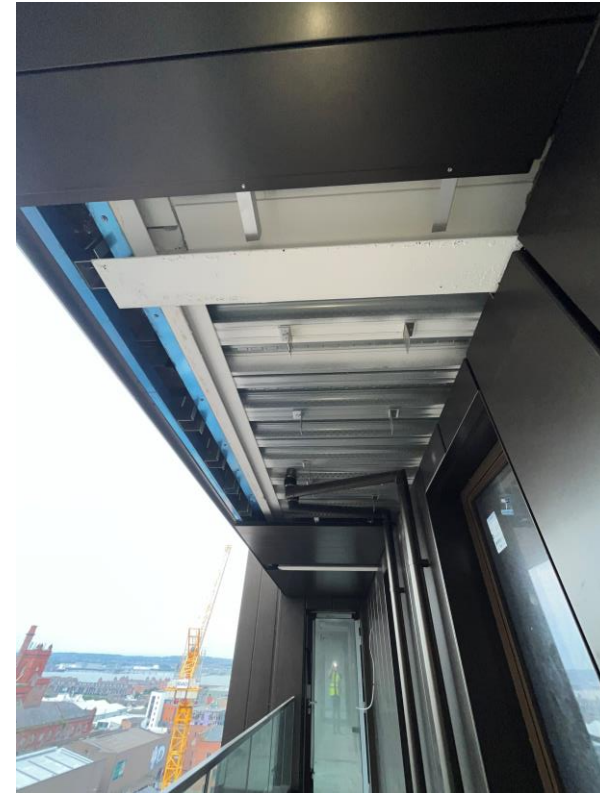
Soffit cladding installation ongoing
