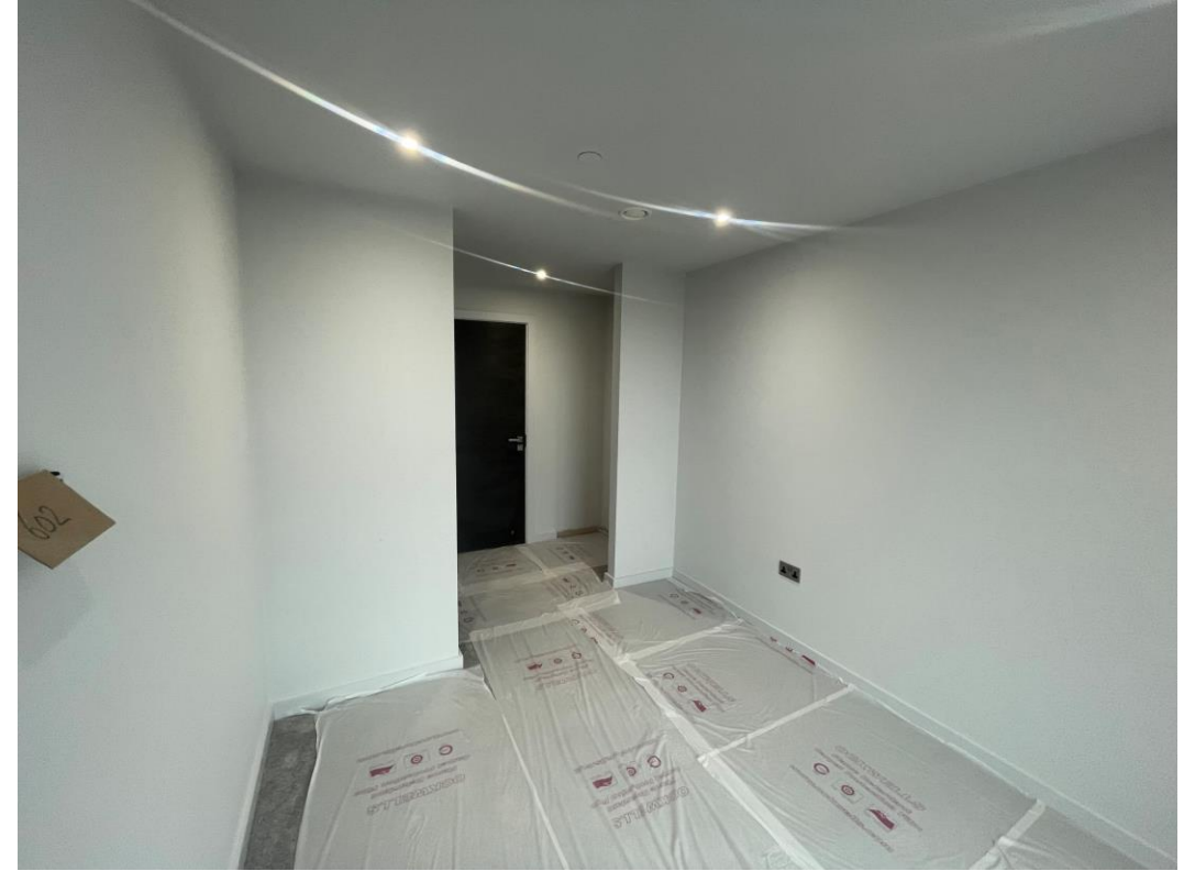
Bedroom carpet installed
