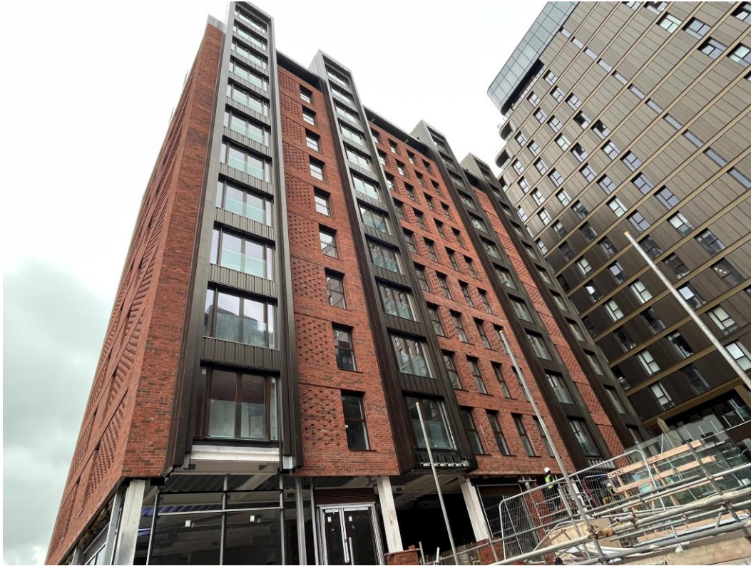
Block B – Brickwork & cladding installation
