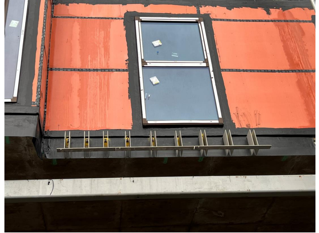
Block D Section A – Masonry Supports
