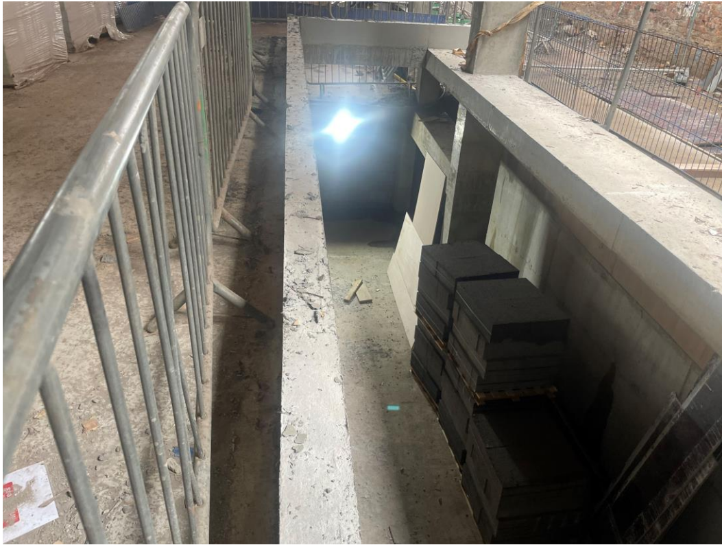
Concrete upstand in place
