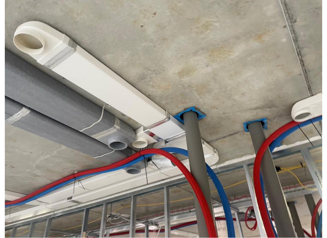
1 st Fix Mechanical ducting ventilation
