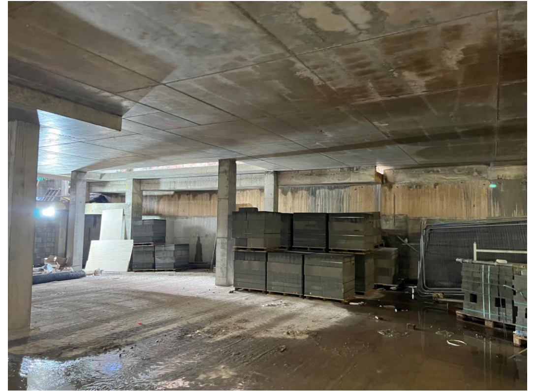
Masonry blockwork on site for installation
