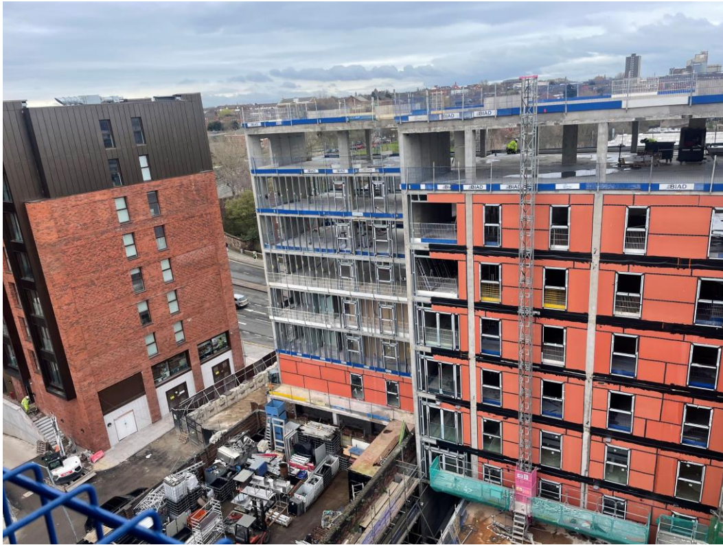
Block D Section A – SFS Installation
