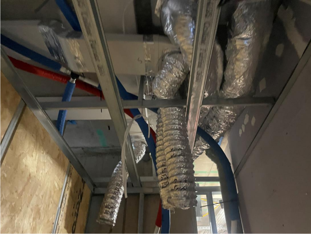
1 st Fix Mechanical ducting ventilation
