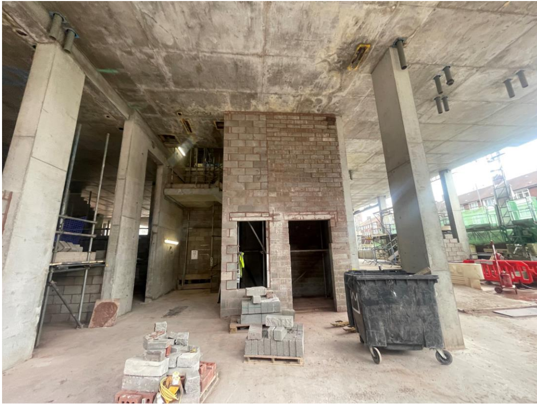
Ground floor blockwork lift shaft
