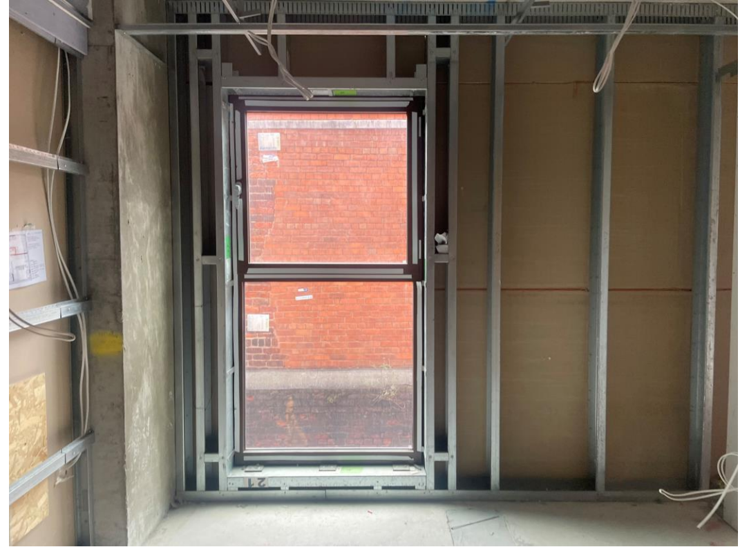
Window installation ongoing
