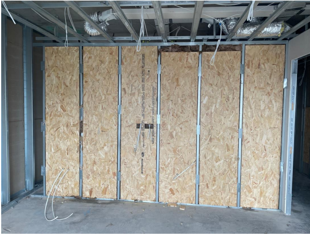
Partitions installation ongoing
