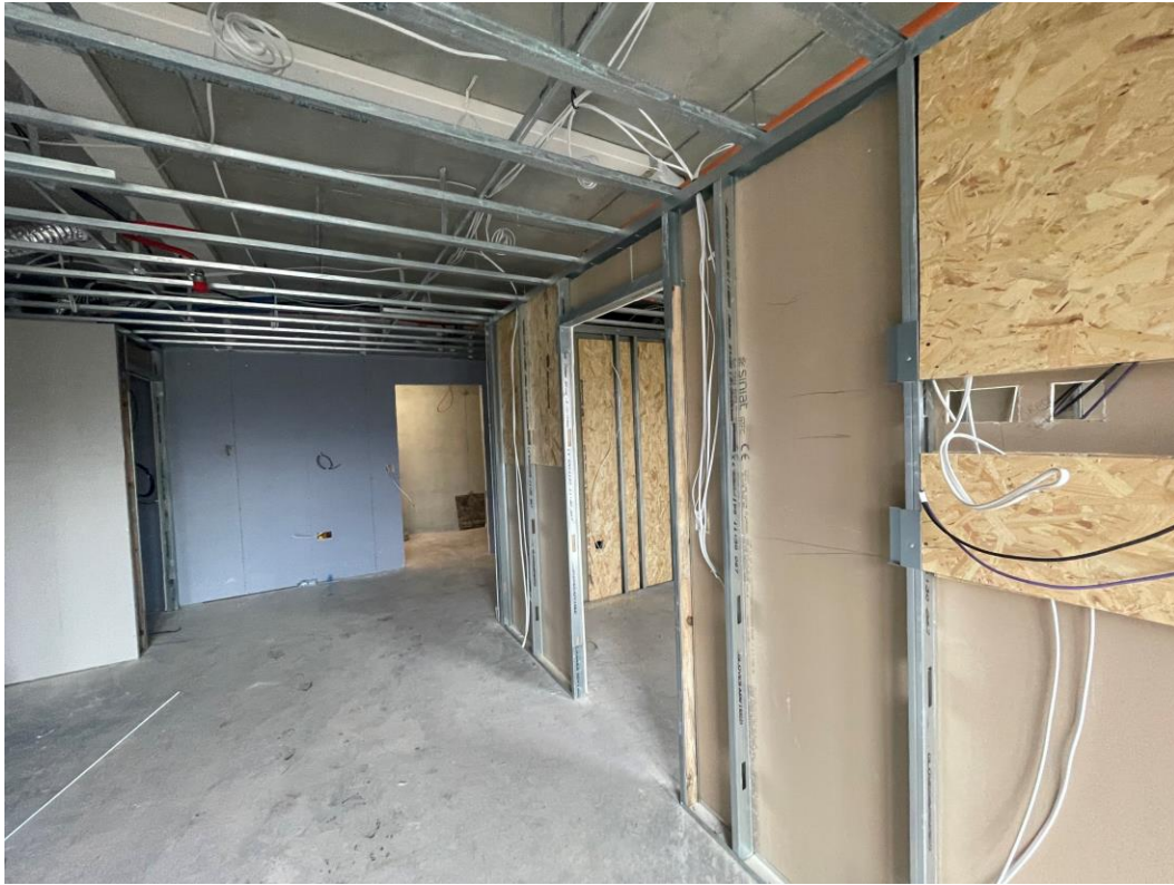
1 st Fix electrical installation commenced
