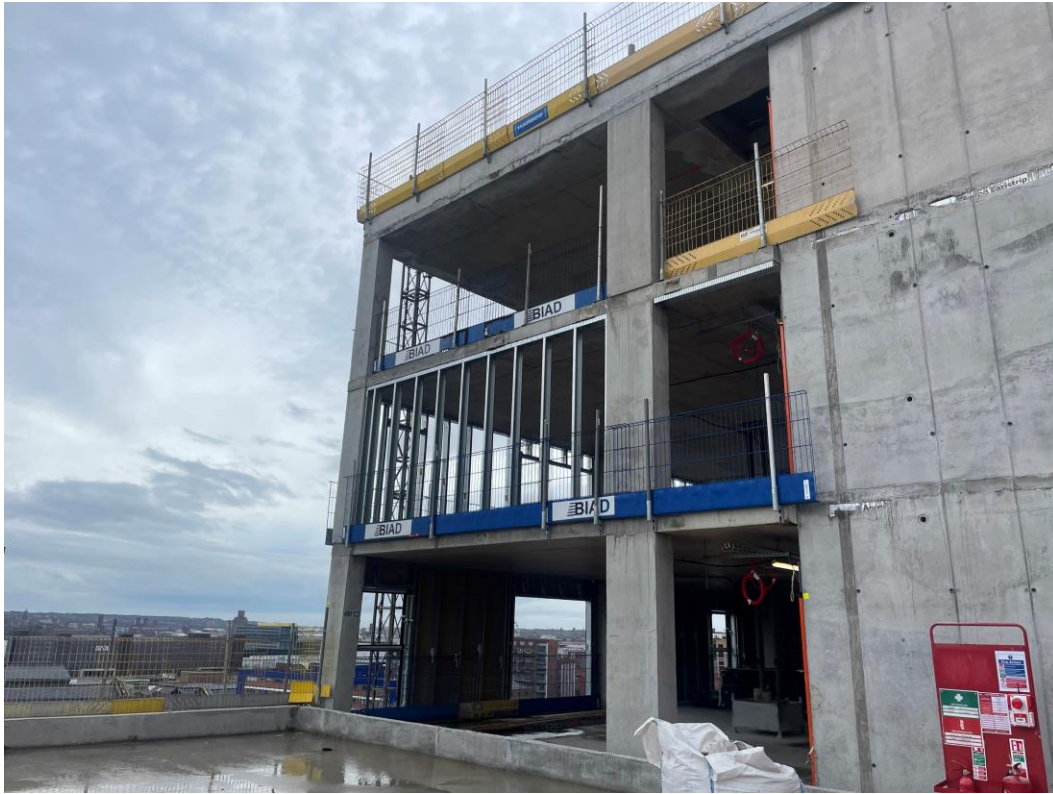
Block D Section A – SFS Installation
