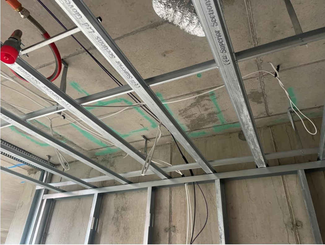
1 st Fix electrical lighting installation commenced
