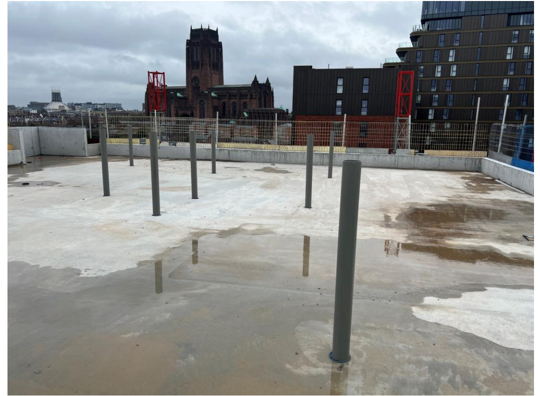
Block D Section A – Roof
