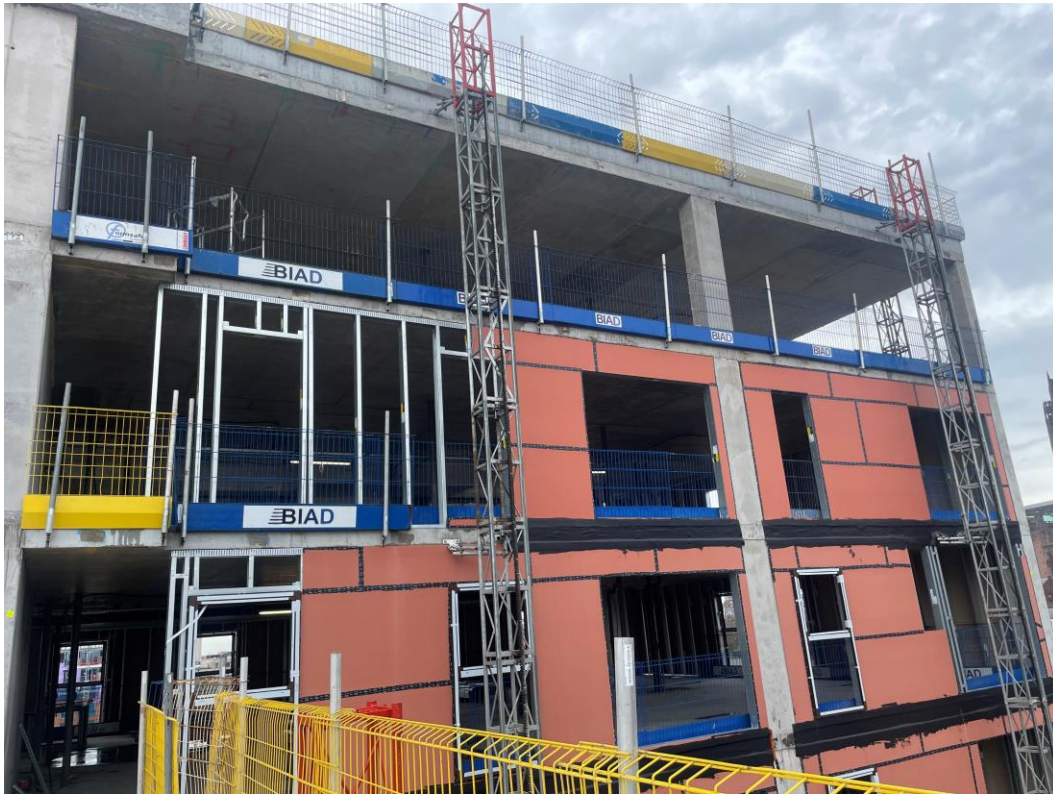
Block D Section A – SFS & Weatherboarding Installation
