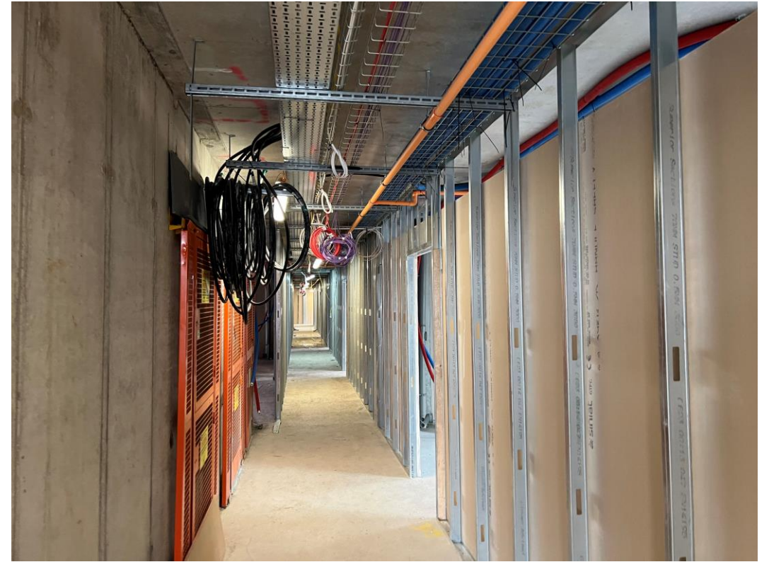
First side partition boarding ongoing
