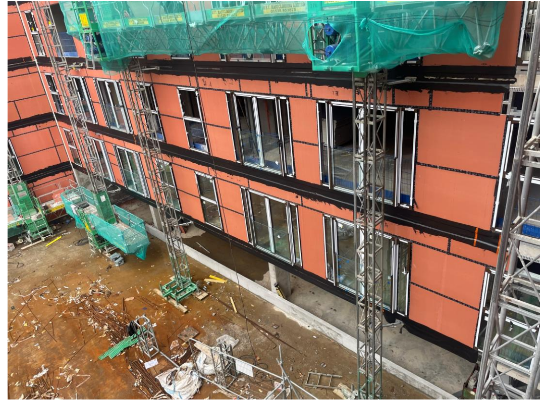
Block D Section C – Glazed balustrade installation
