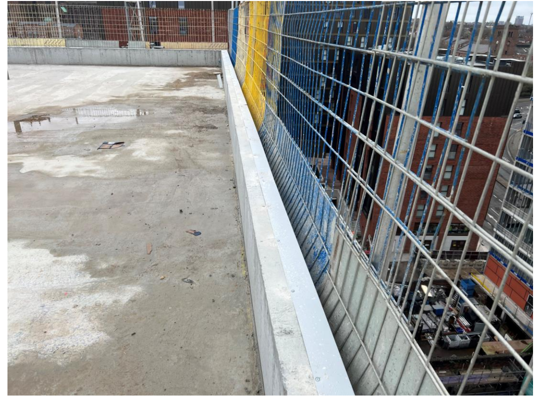
Block D Section B – Roof works
