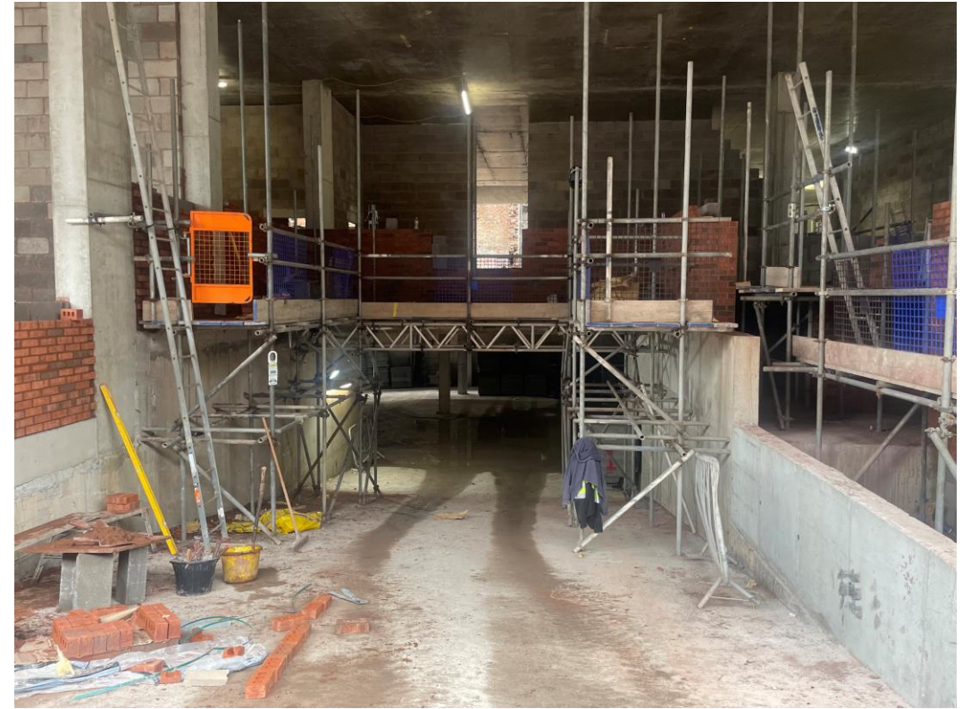
Ground floor brickwork walls
