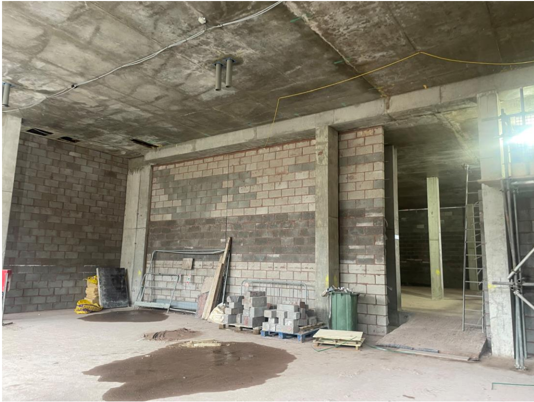
Ground floor blockwork wall
