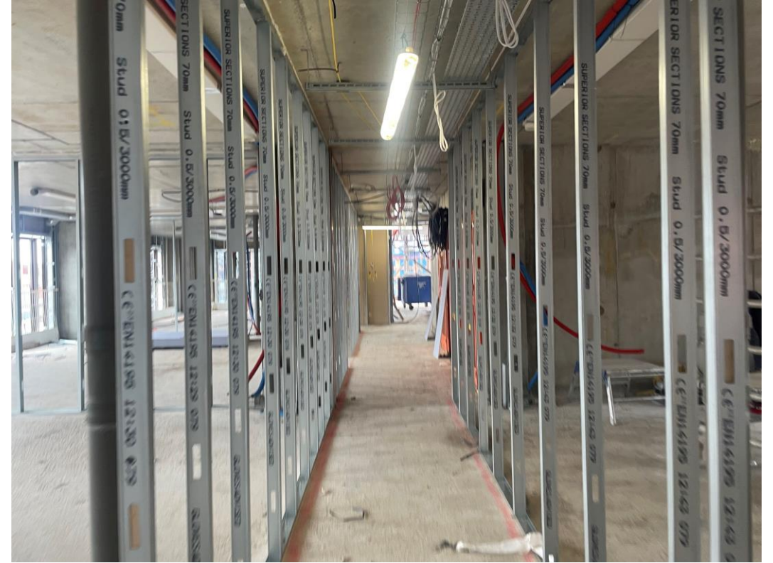
Metal partition frame work installation commenced
