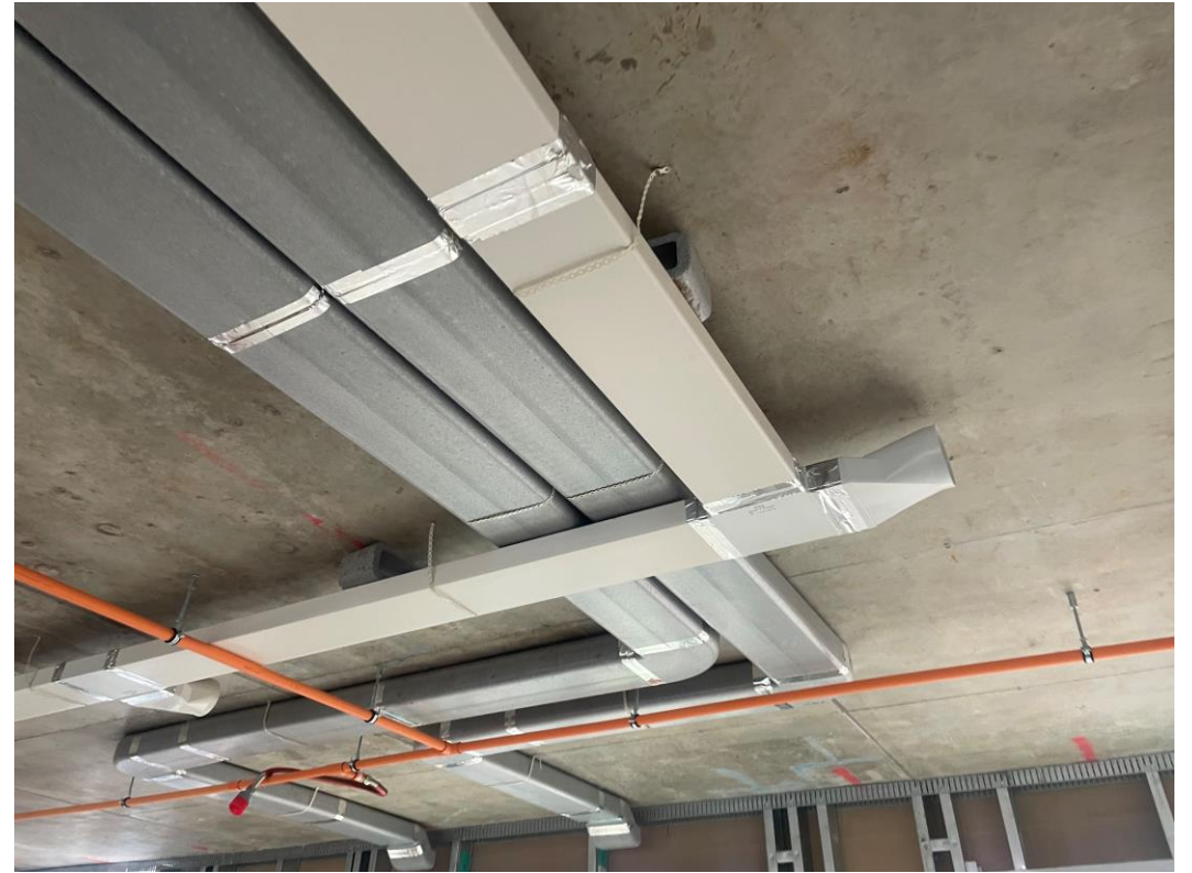
1 st Fix Mechanical ducting ventilation
