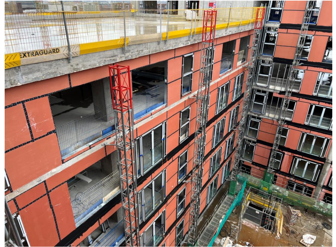
Block D Section C – SFS & Weatherboarding Installation
