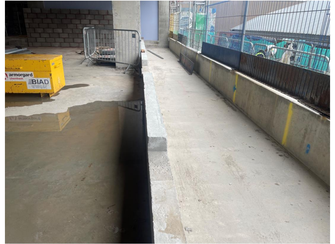
Section C - Concrete upstand in place for curtain walling
