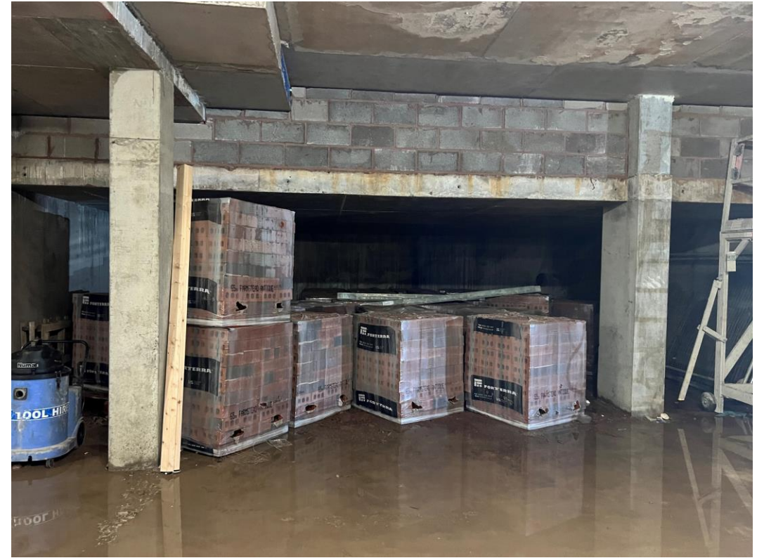
Facing brick stored
