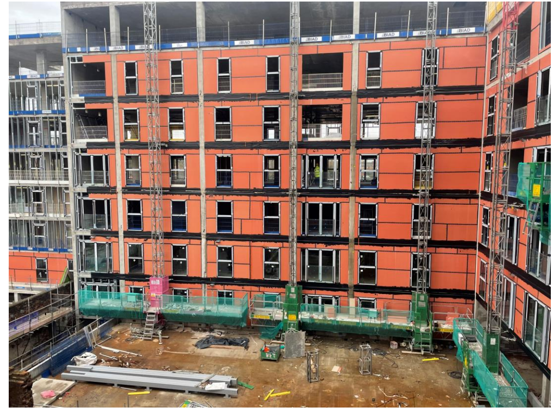
Block D Section B – SFS & Weatherboarding Installation
