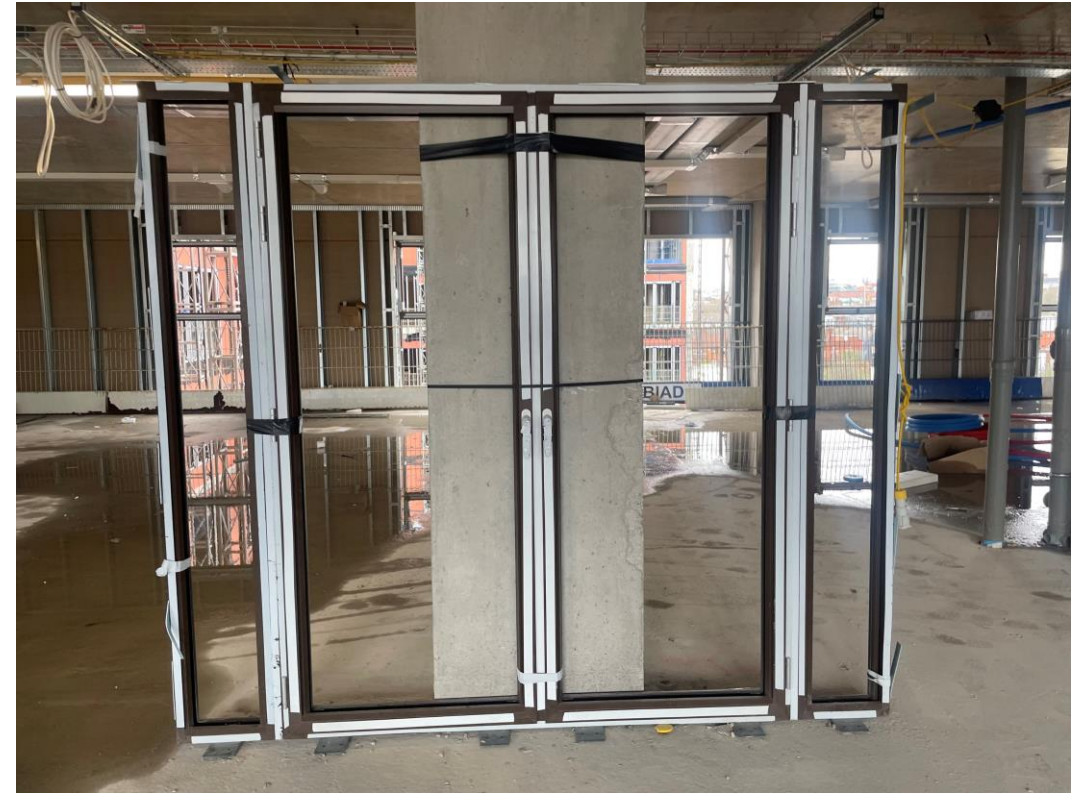
Window frames on site for installation
