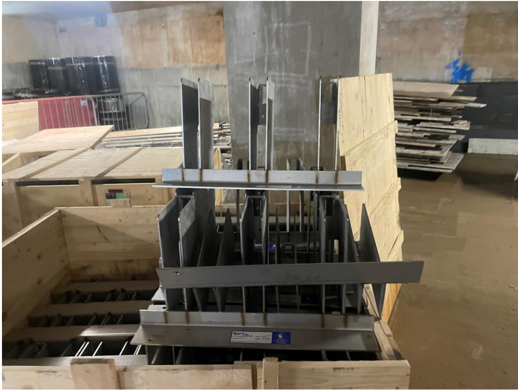
Masonry supports on site for installation
