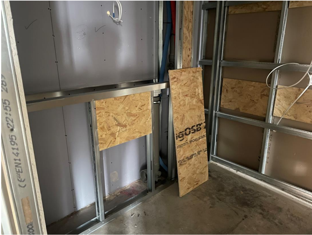
Metal IPS installation commenced
