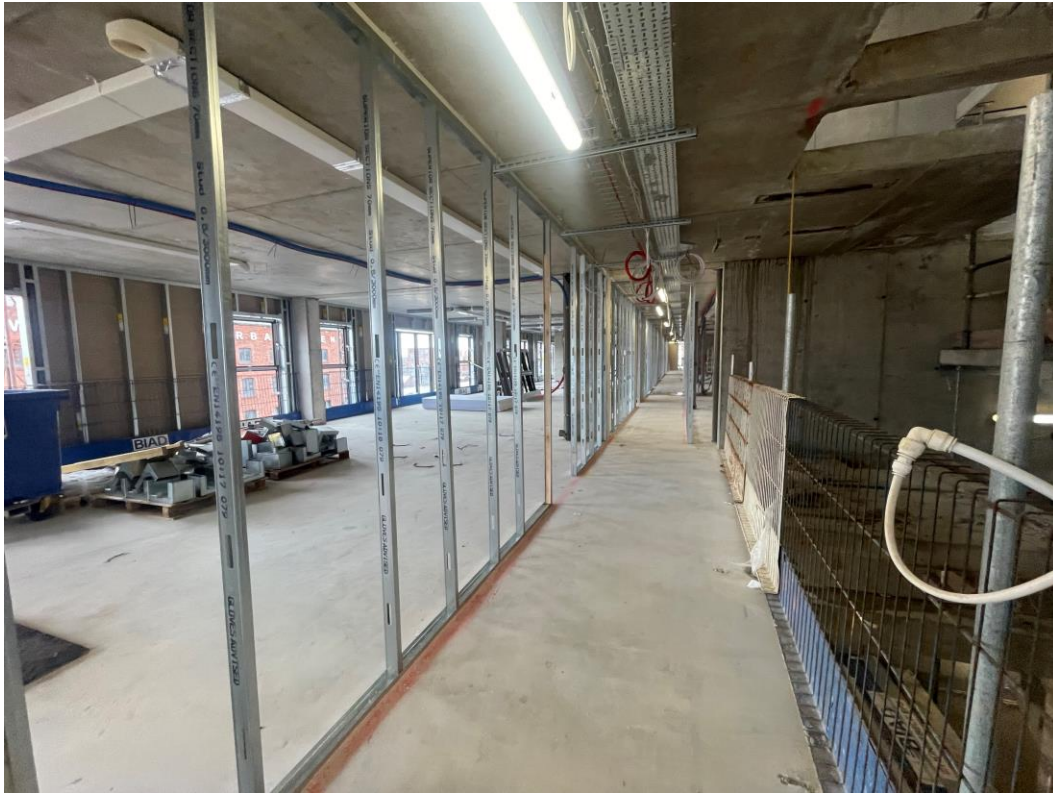
Metal partition frame work installation commenced
