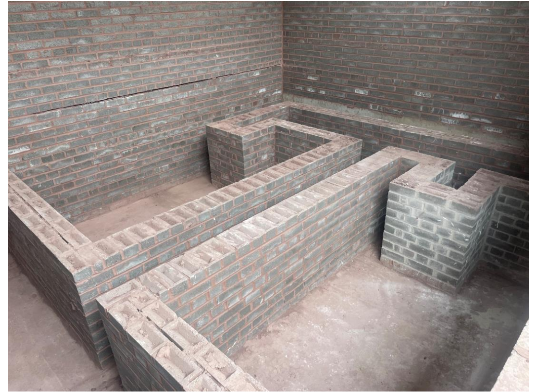
Substation substructure brickwork
