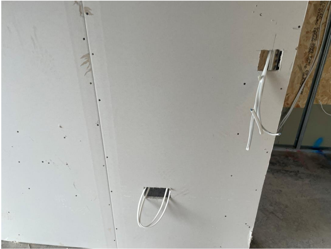
1 st Fix electrical installation commenced
