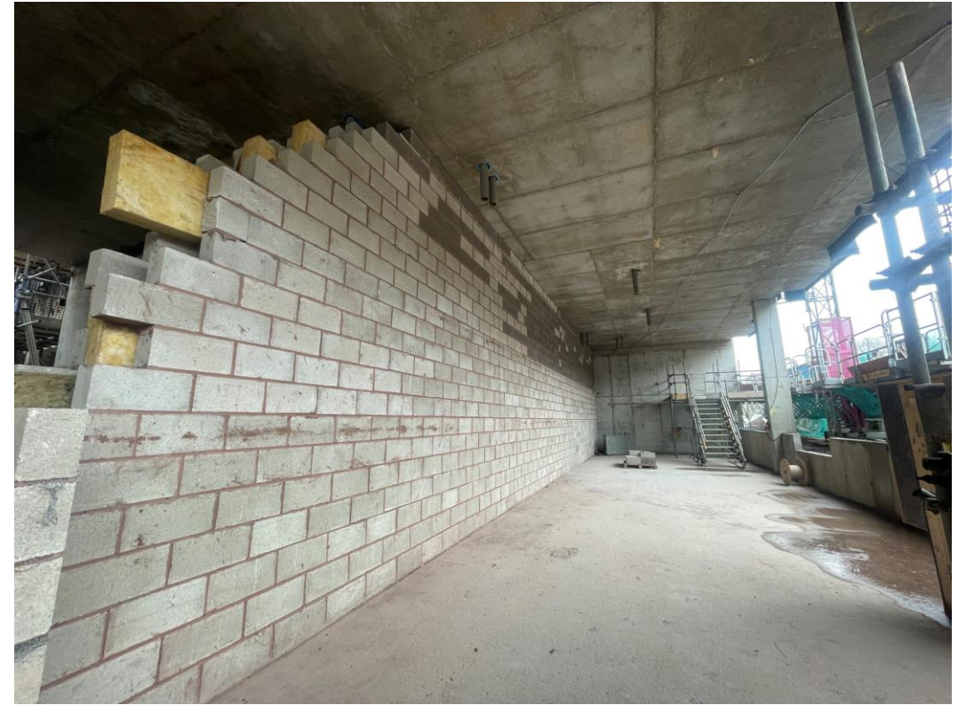
Ground floor blockwork wall
