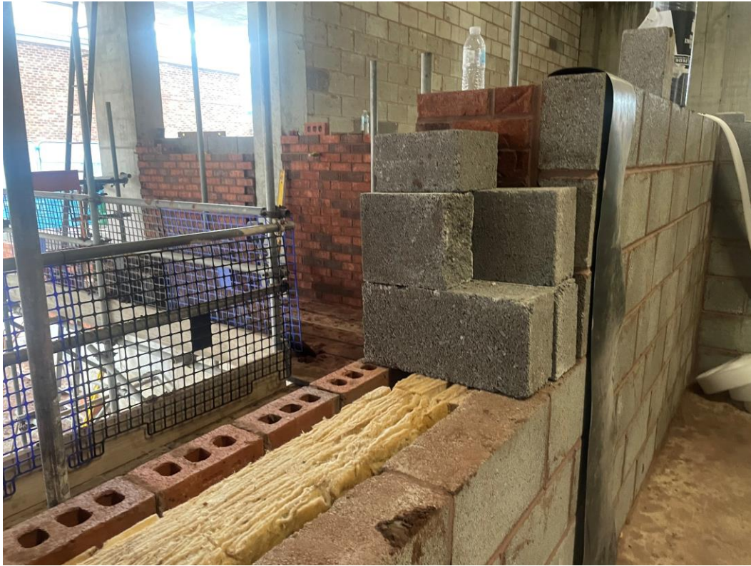
Ground floor insulated cavity wall
