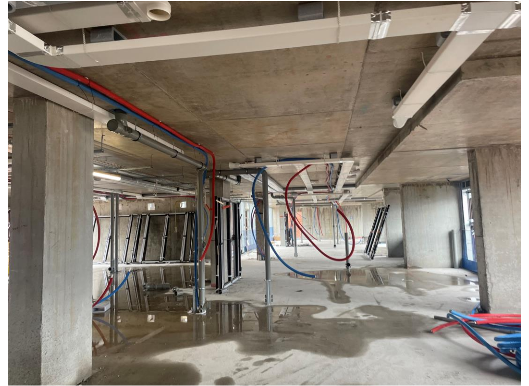
1st Fix water distribution to apartments
