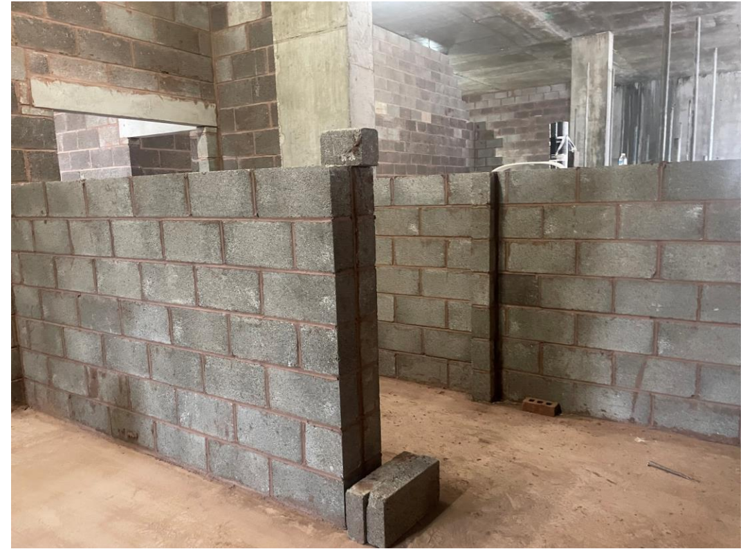
Ground floor blockwork wall
