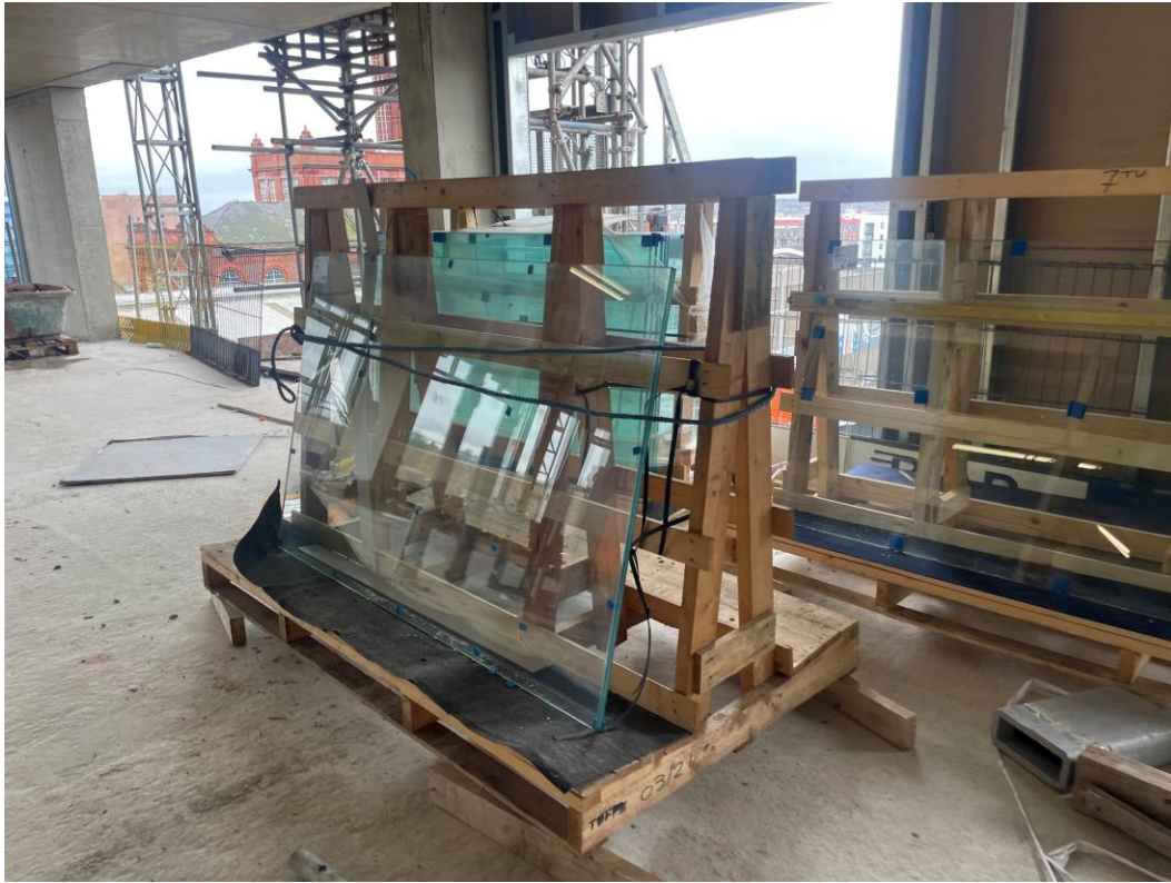
Glazing units on site for installation
