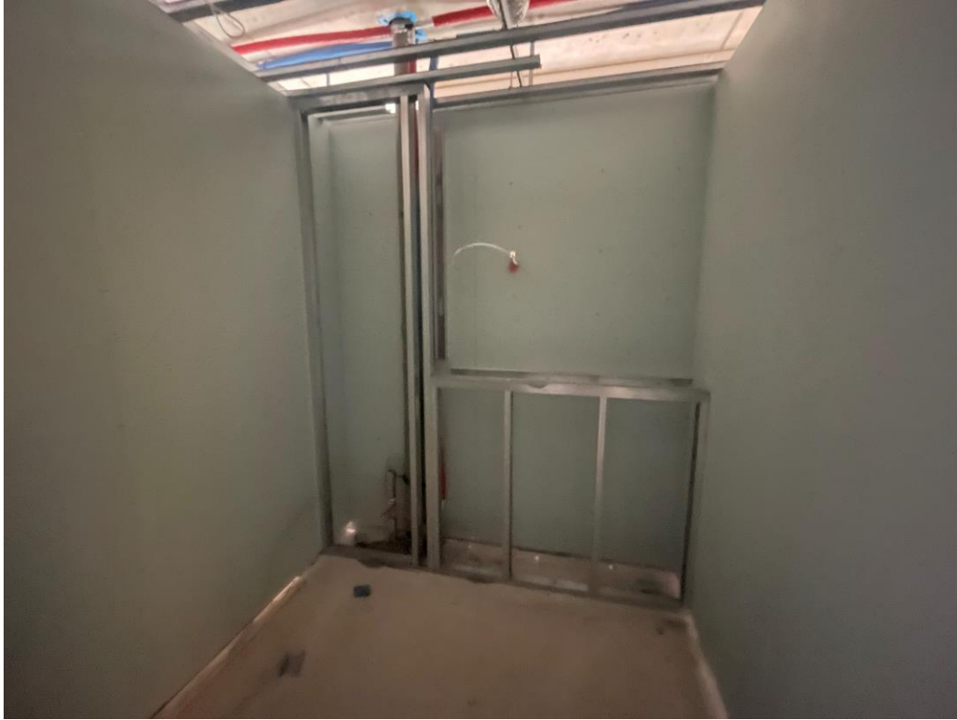
Metal IPS installation commenced
