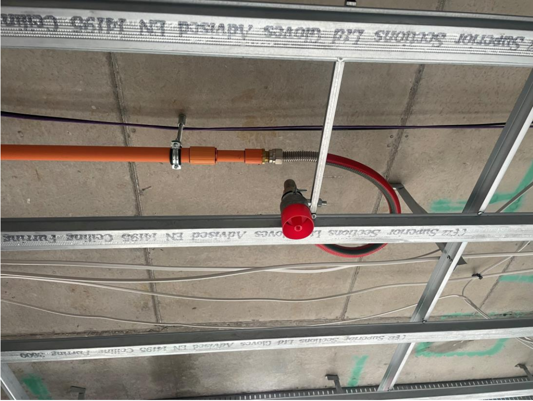
Sprinkler system installation commenced
