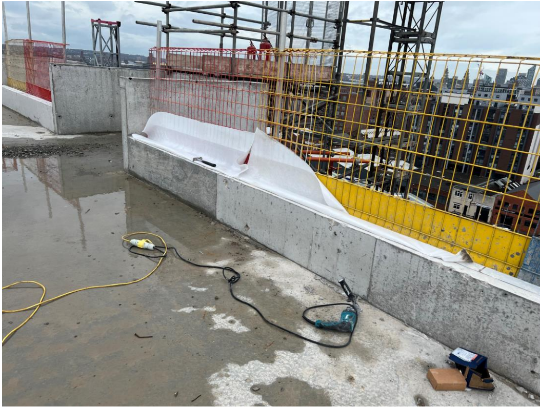
Block D Section A – Roof works
