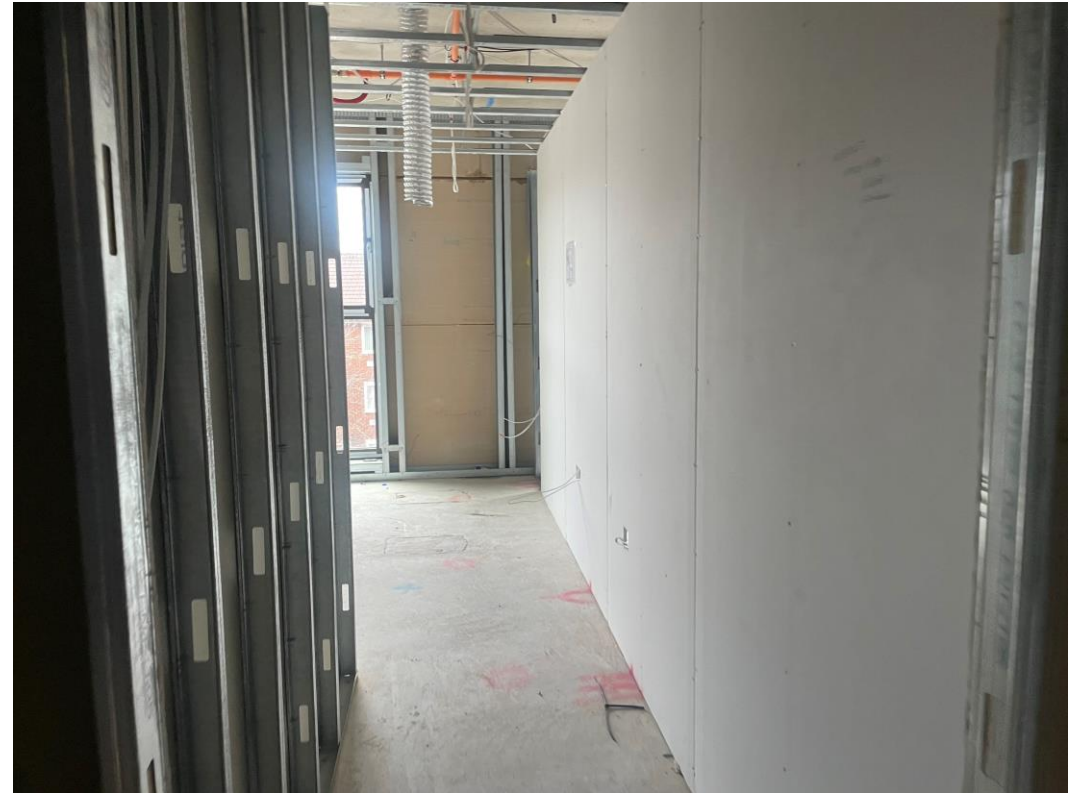
First side partition boarding ongoing
