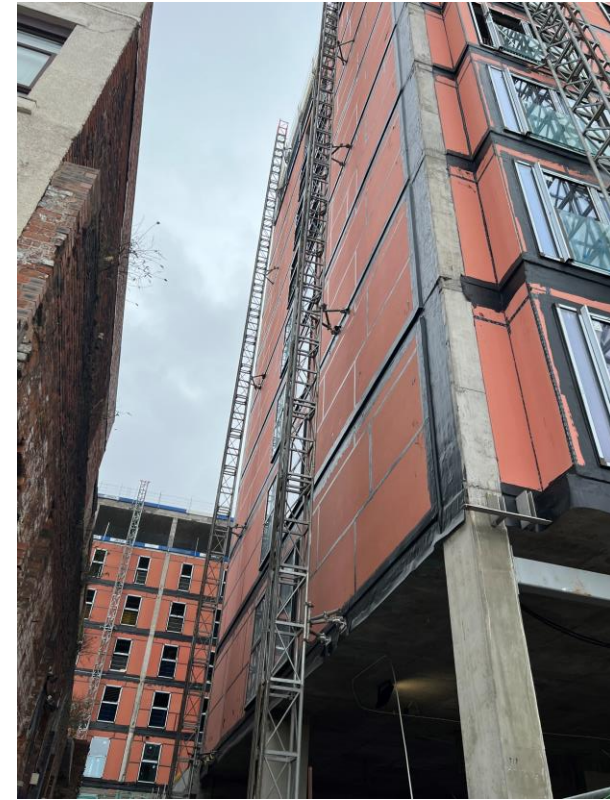
Block D Section A – Viewed from Site Compound
