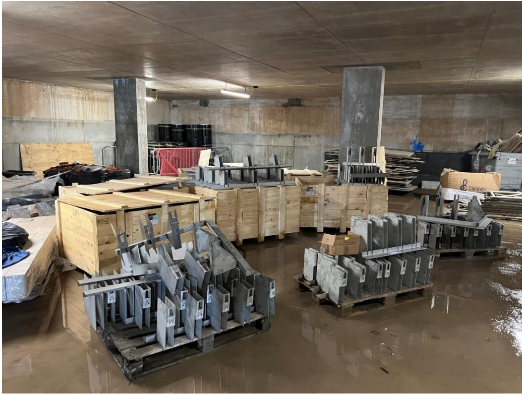
Masonry supports on site for installation
