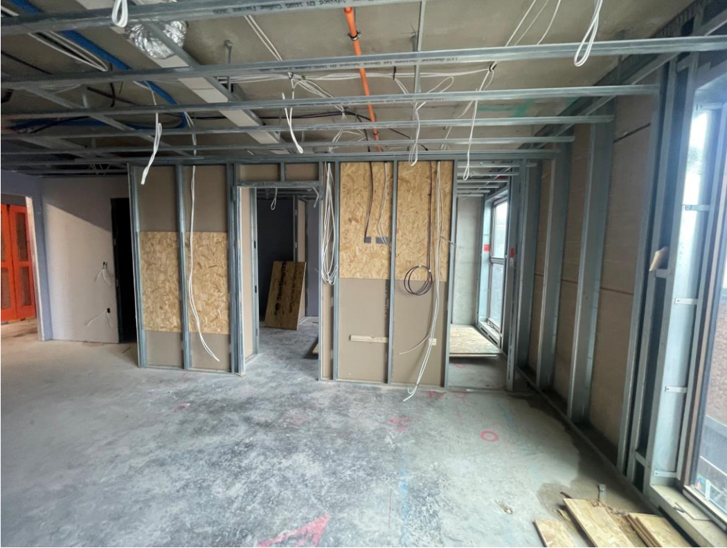
1 st Fix electrical installation commenced
