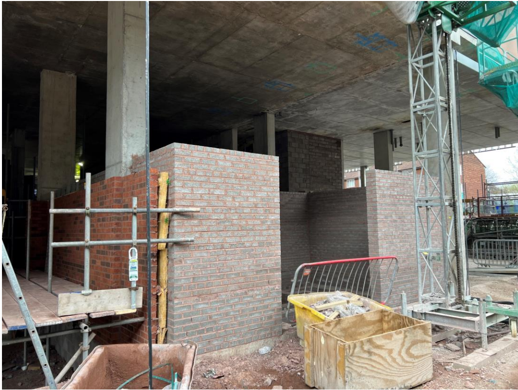
Substation brickwork walls
