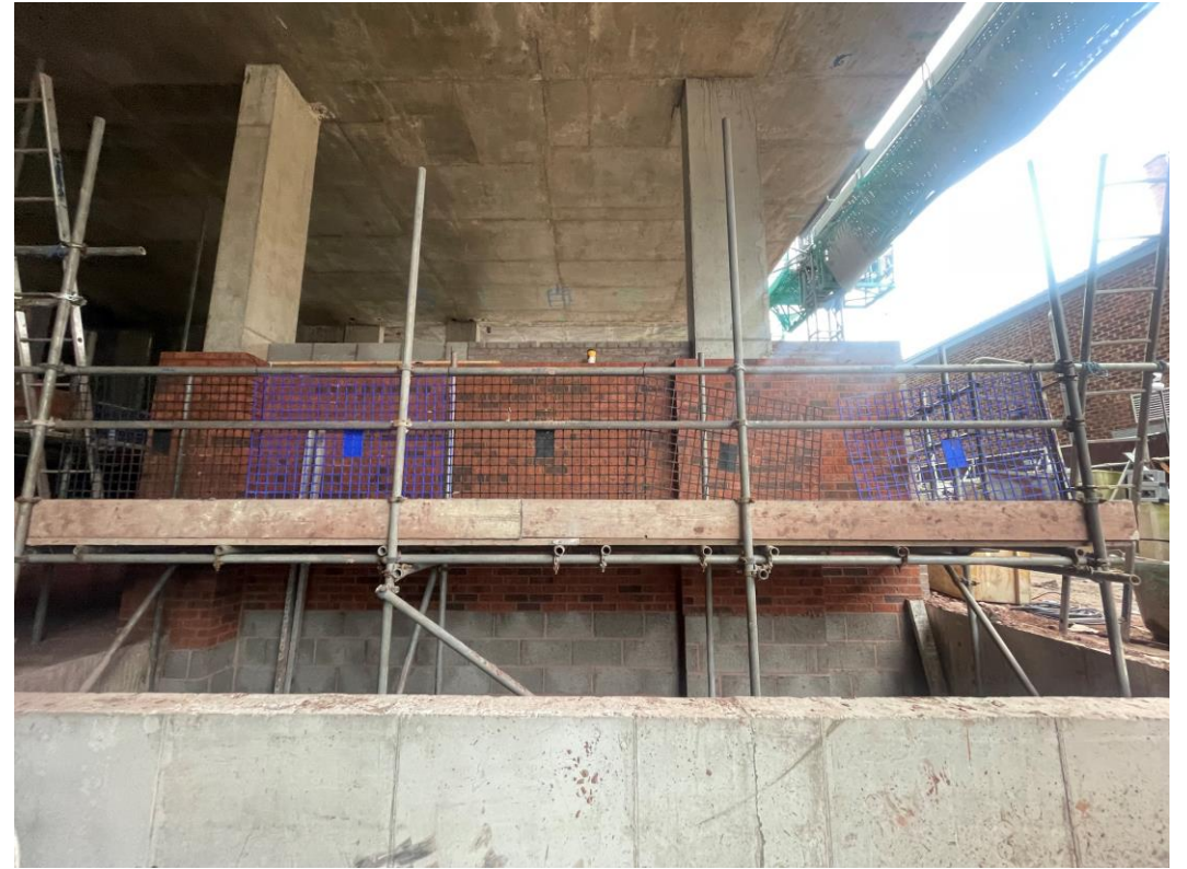
Ground floor brickwork walls
