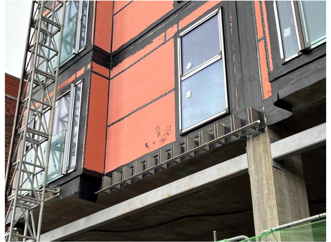
Block D Section A – Masonry Supports
