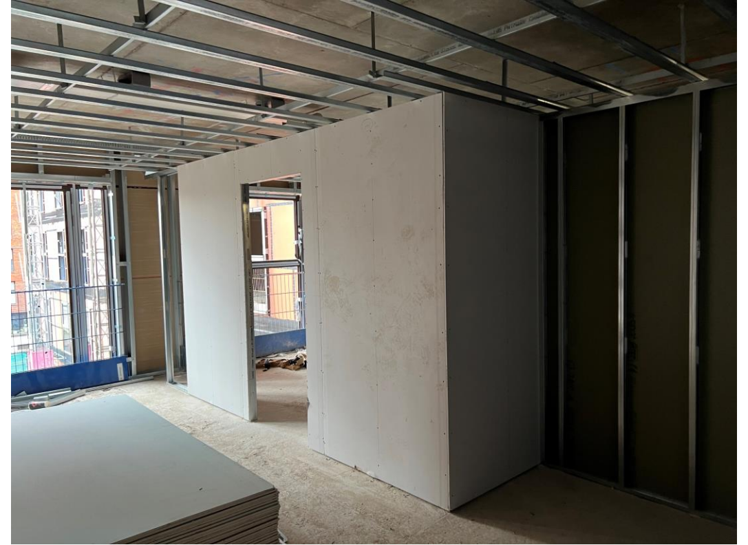
First side partition boarding ongoing
