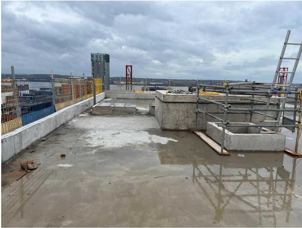
Block D Section B – Roof
