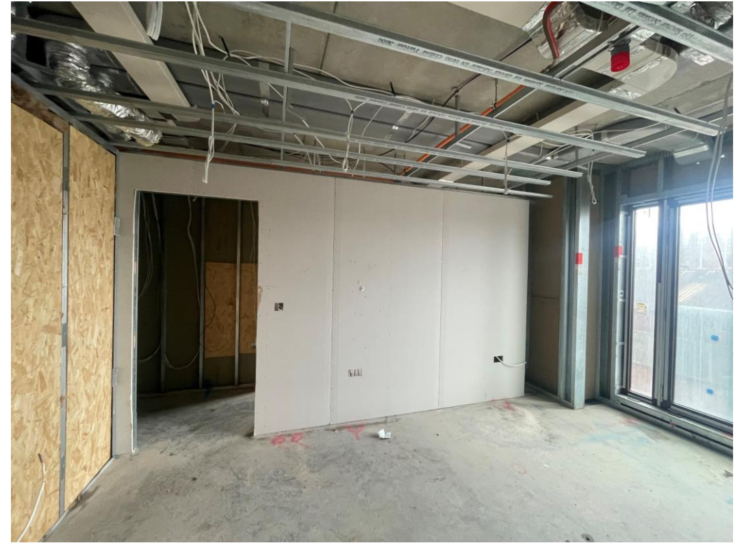
First side partition boarding ongoing
