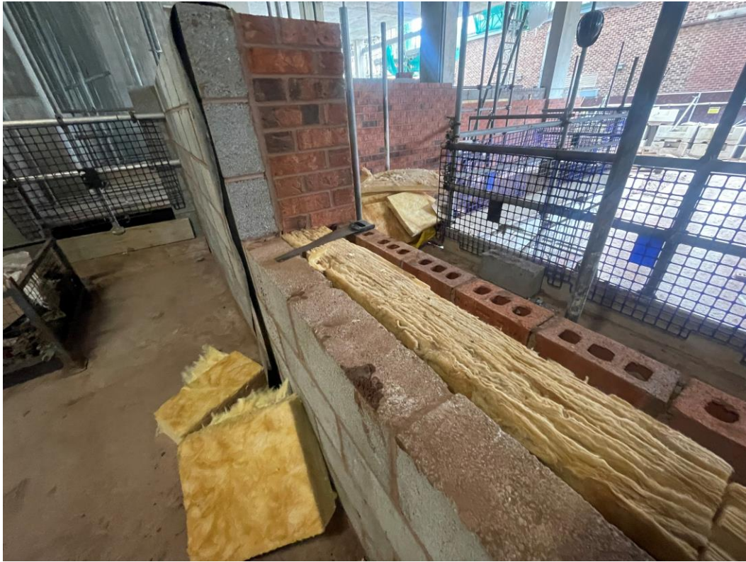
Ground floor insulated cavity wall
