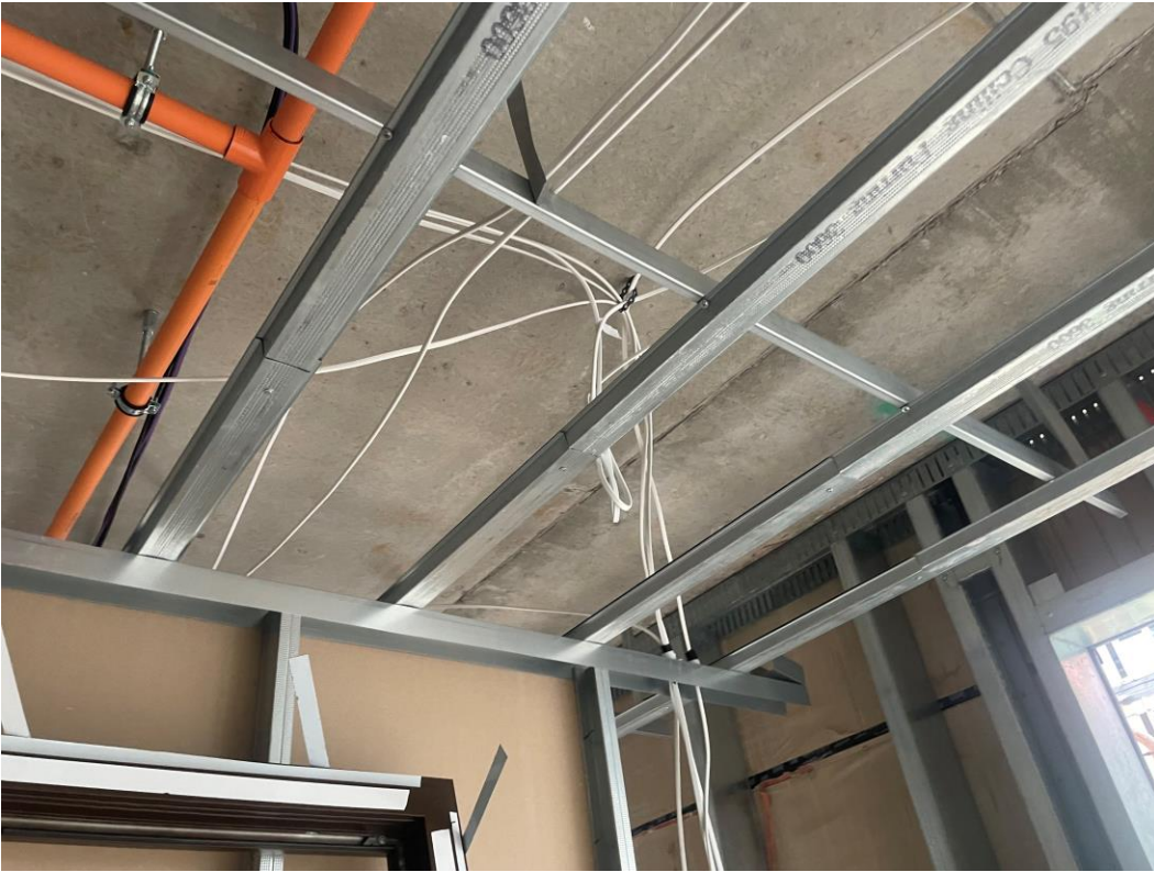
1 st Fix electrical lighting installation commenced
