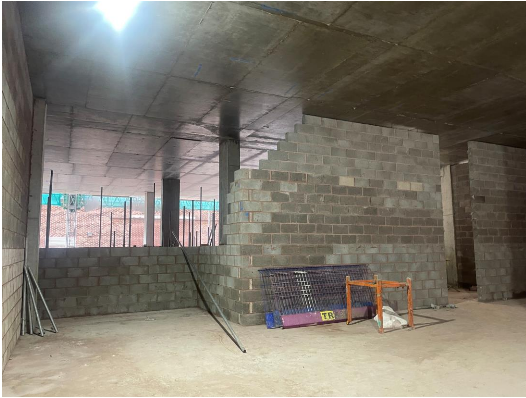
Ground floor blockwork walls
