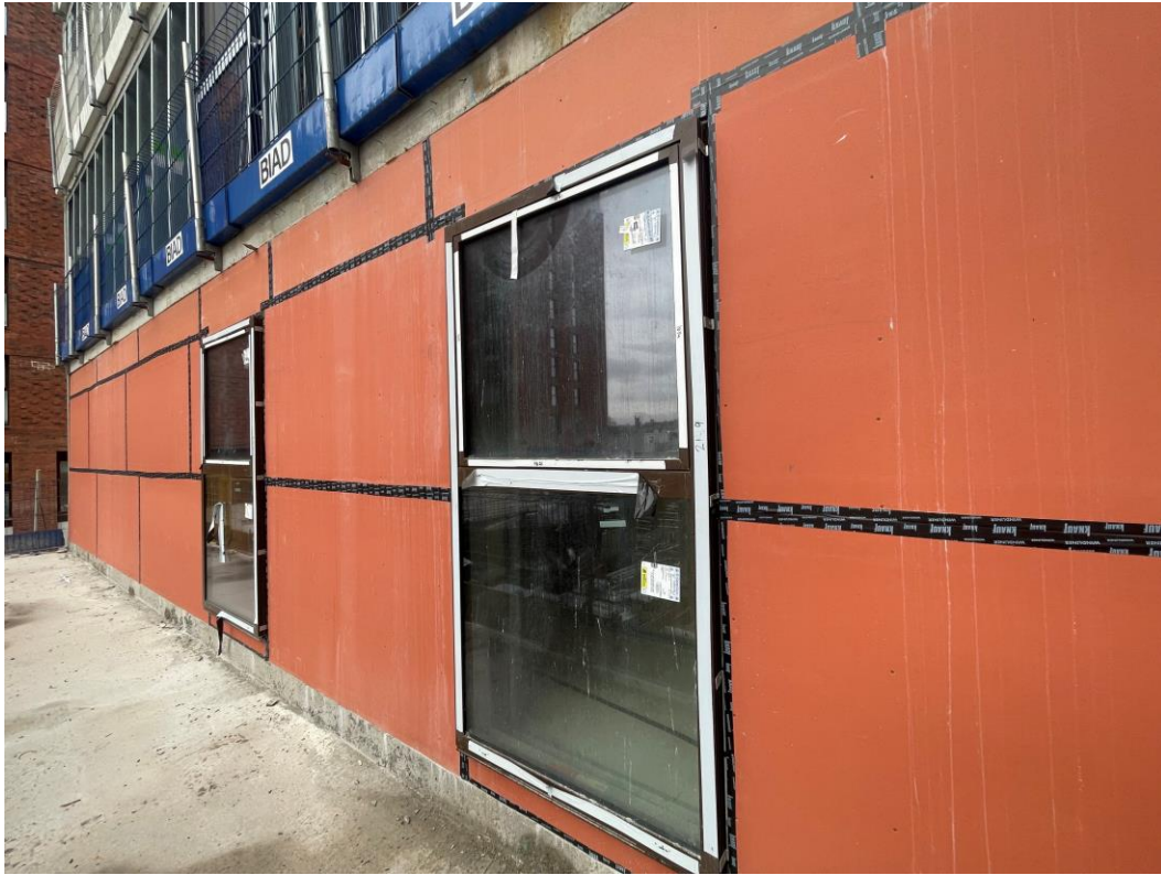
Block D Section A – Window units
