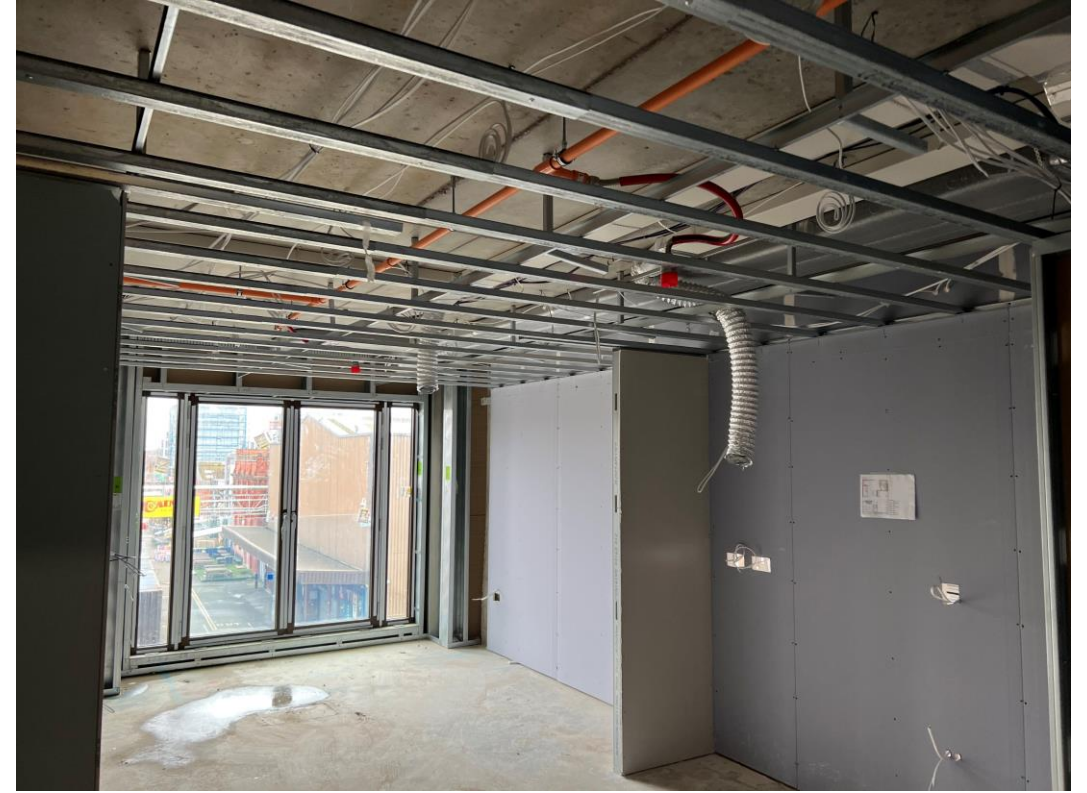
Metal ceiling grid installation commenced
