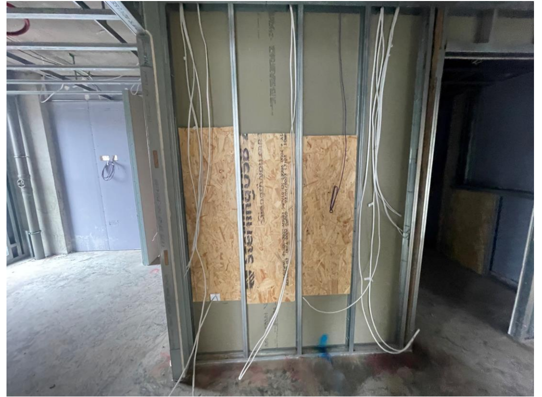
1 st Fix electrical installation commenced
