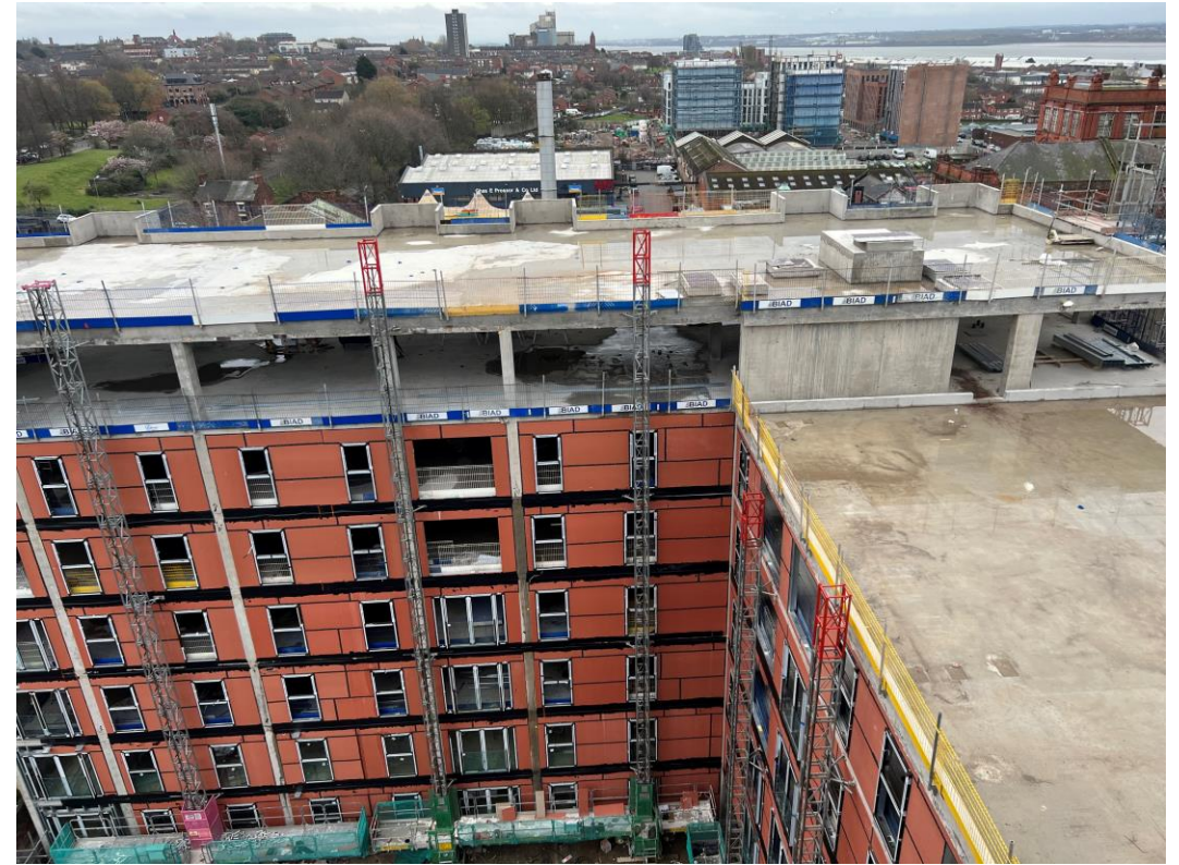
Block D Section B – Roof
