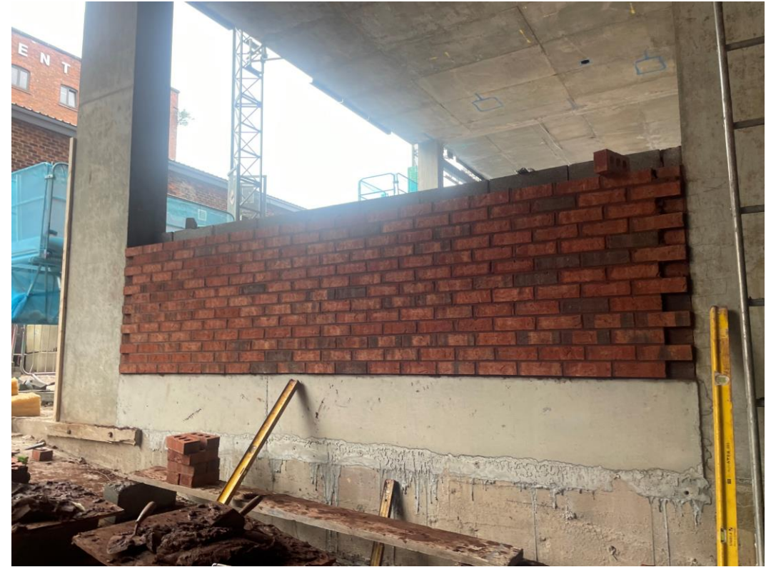
Ground floor brickwork walls
