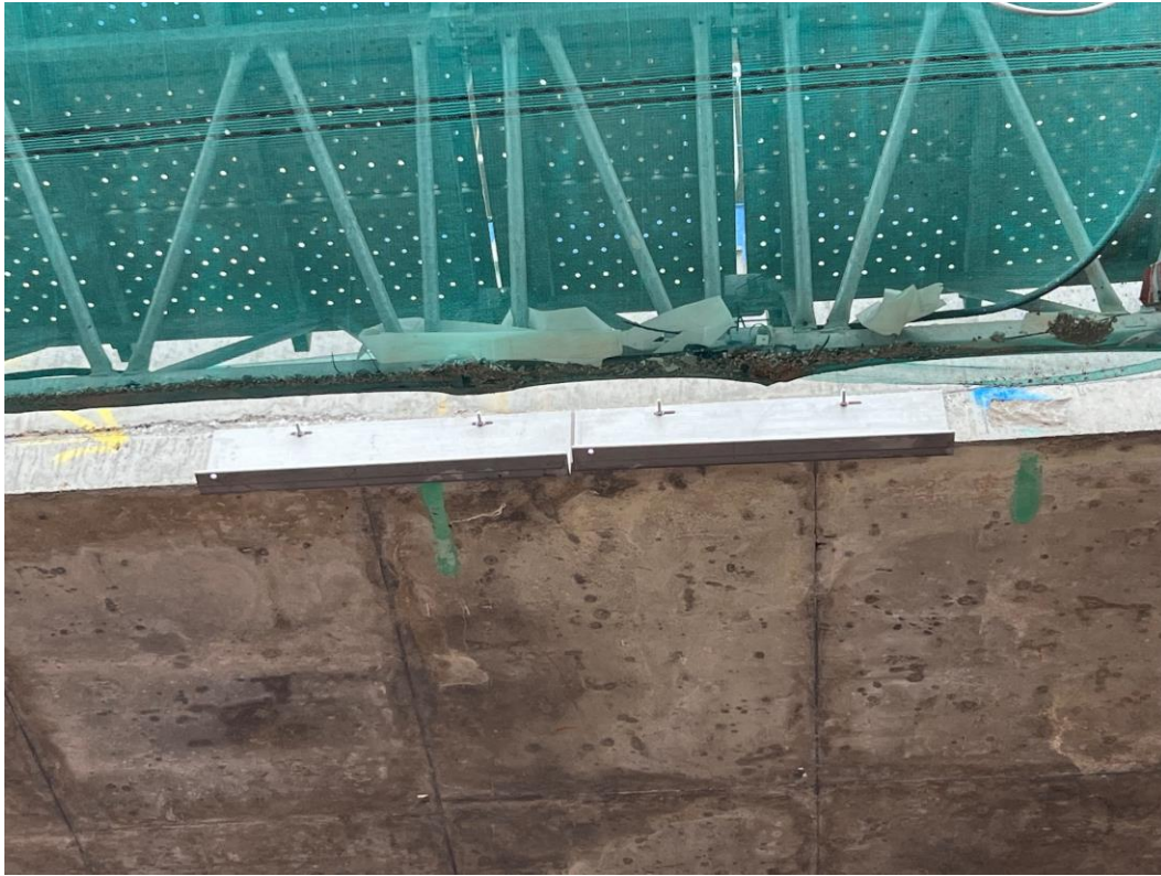
Block D Section A – Masonry Supports
