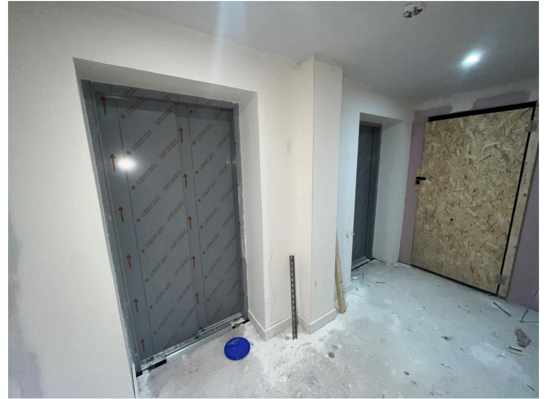
1 st coat decoration to walls & ceilings
