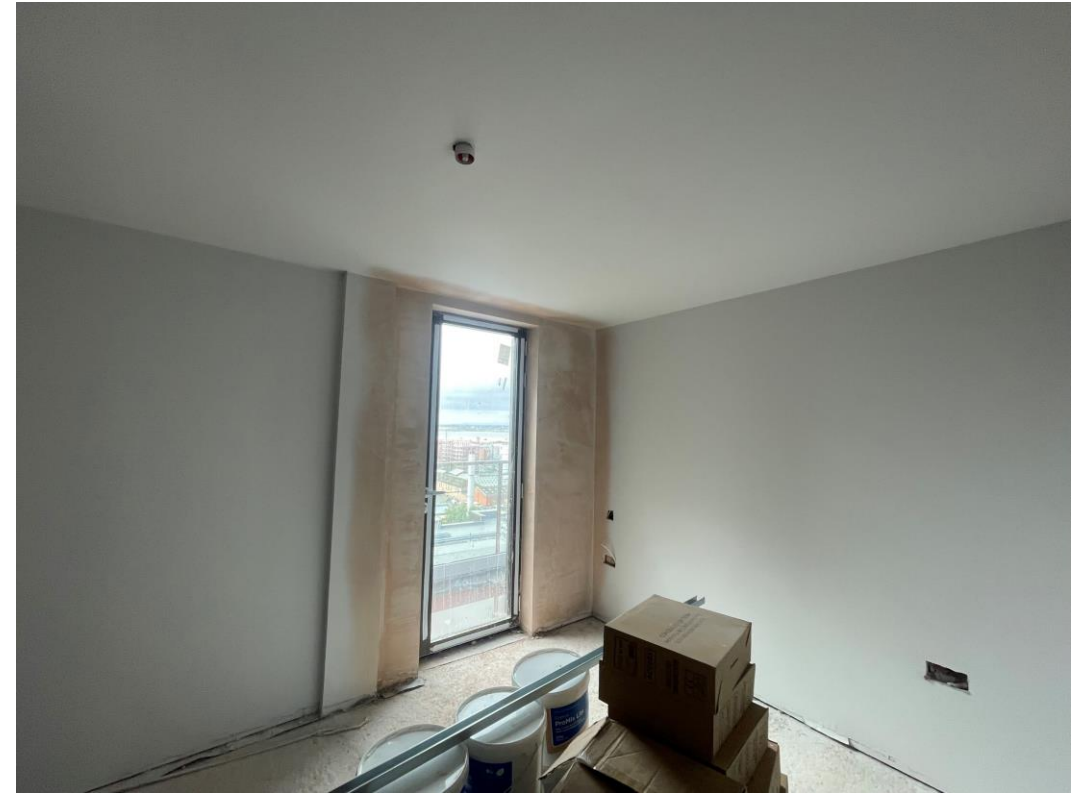
2 nd Coat decoration walls & ceilings
