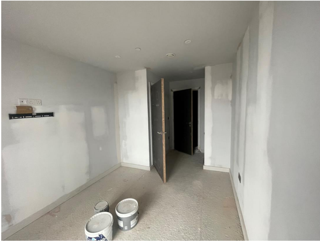
Bedroom finishes ongoing
