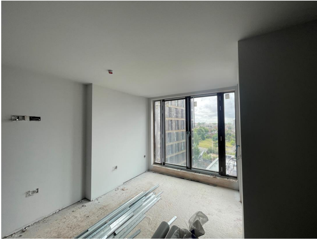
Lounge finishes ongoing
