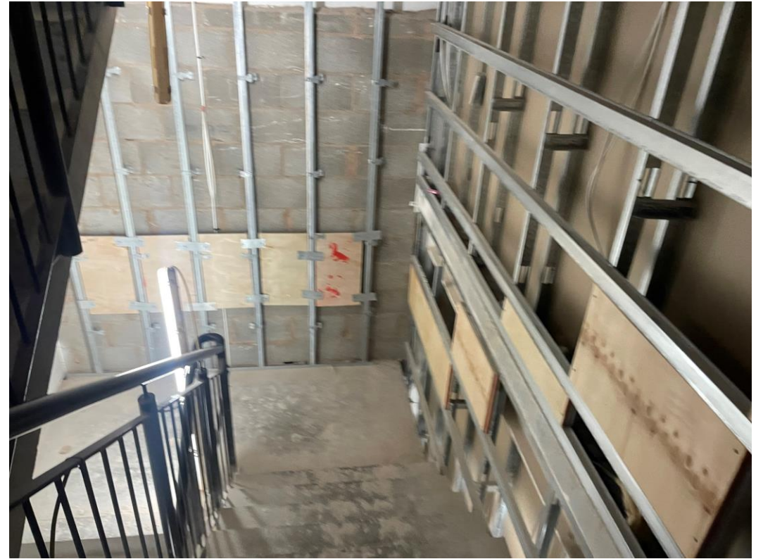
Staircase pattress installed
