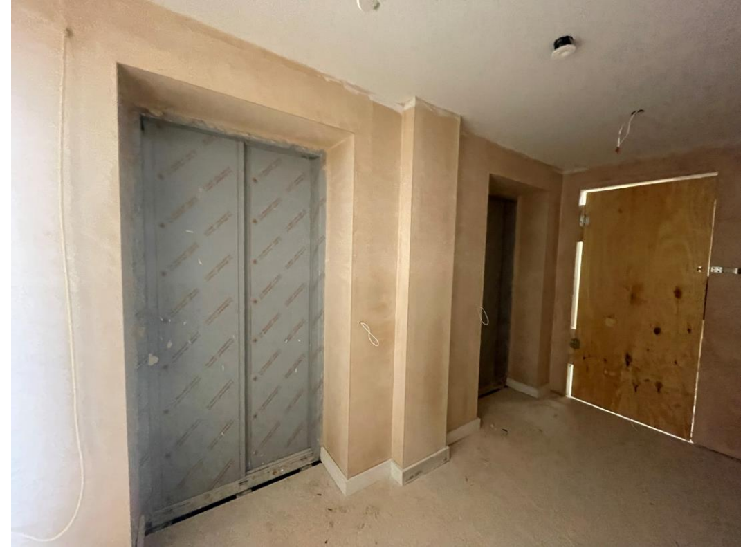
Walls & ceiling to lift areas plastered
