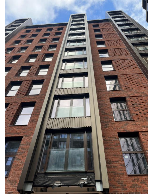
Block B – Brickwork & cladding installation
