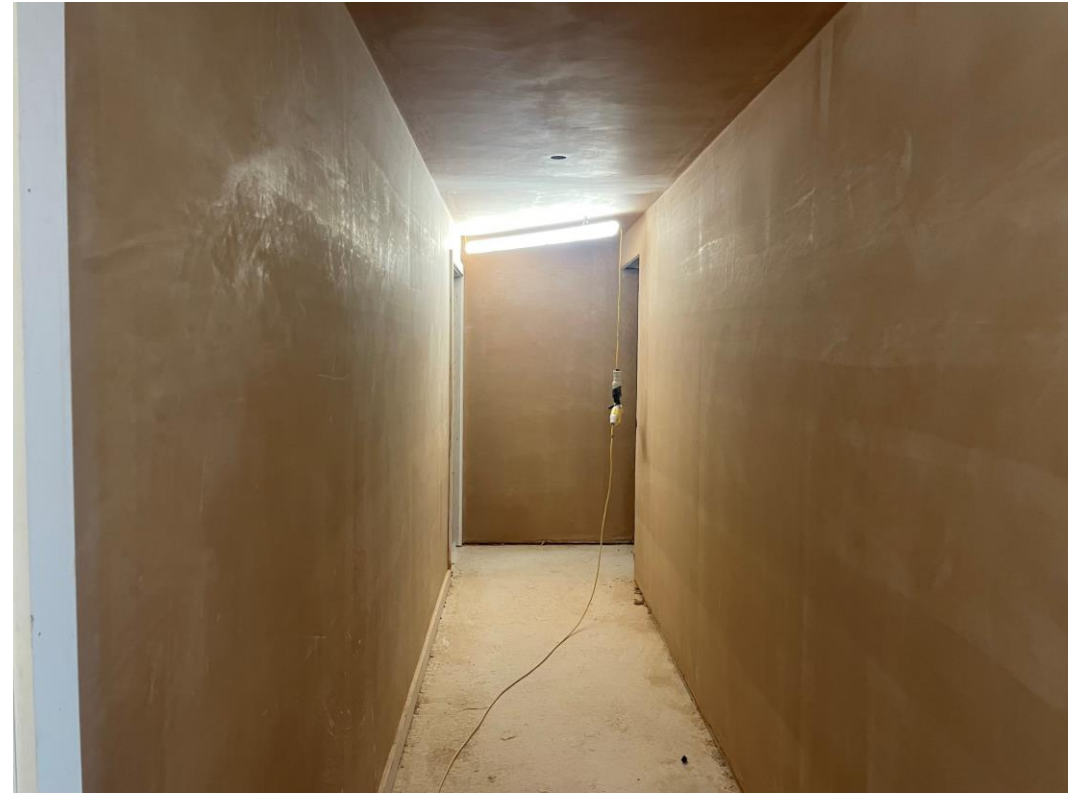
Circulation areas walls & ceilings plastered
