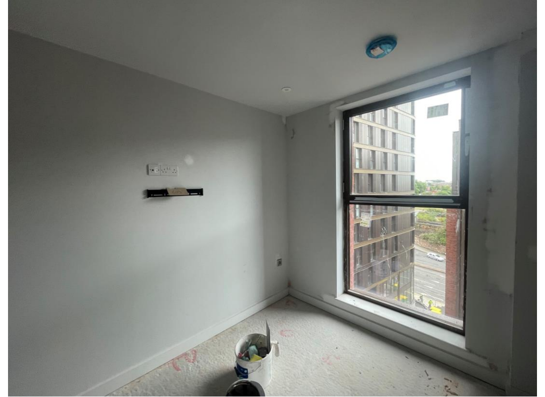
2 nd Coat wall & ceiling decoration to bedrooms
