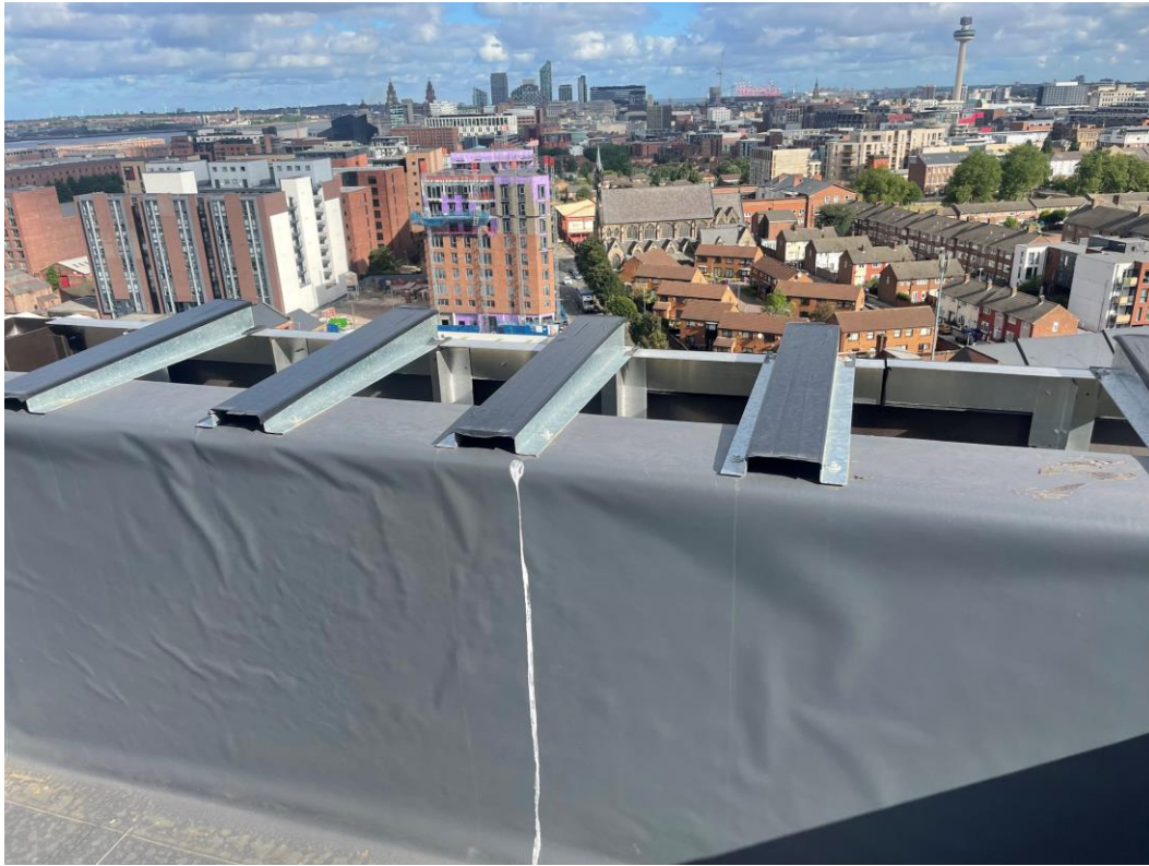
Cladding capping details installation ongoing
