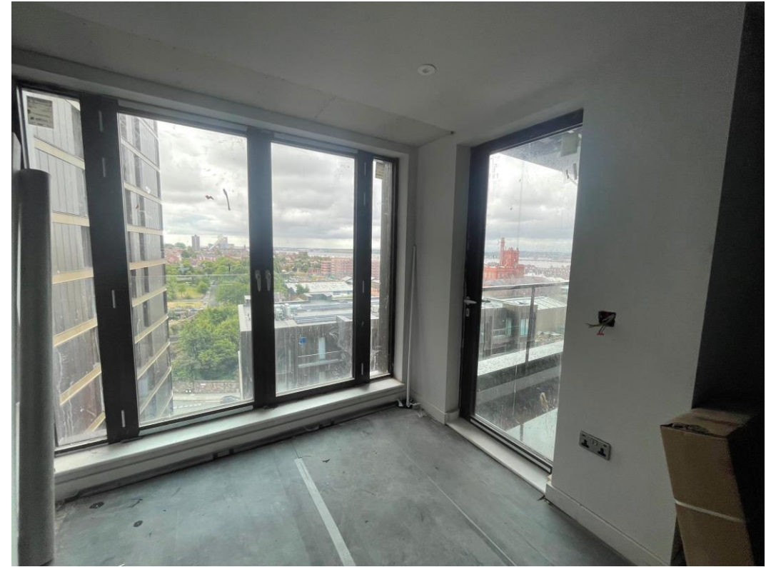
Lounge finishes ongoing
