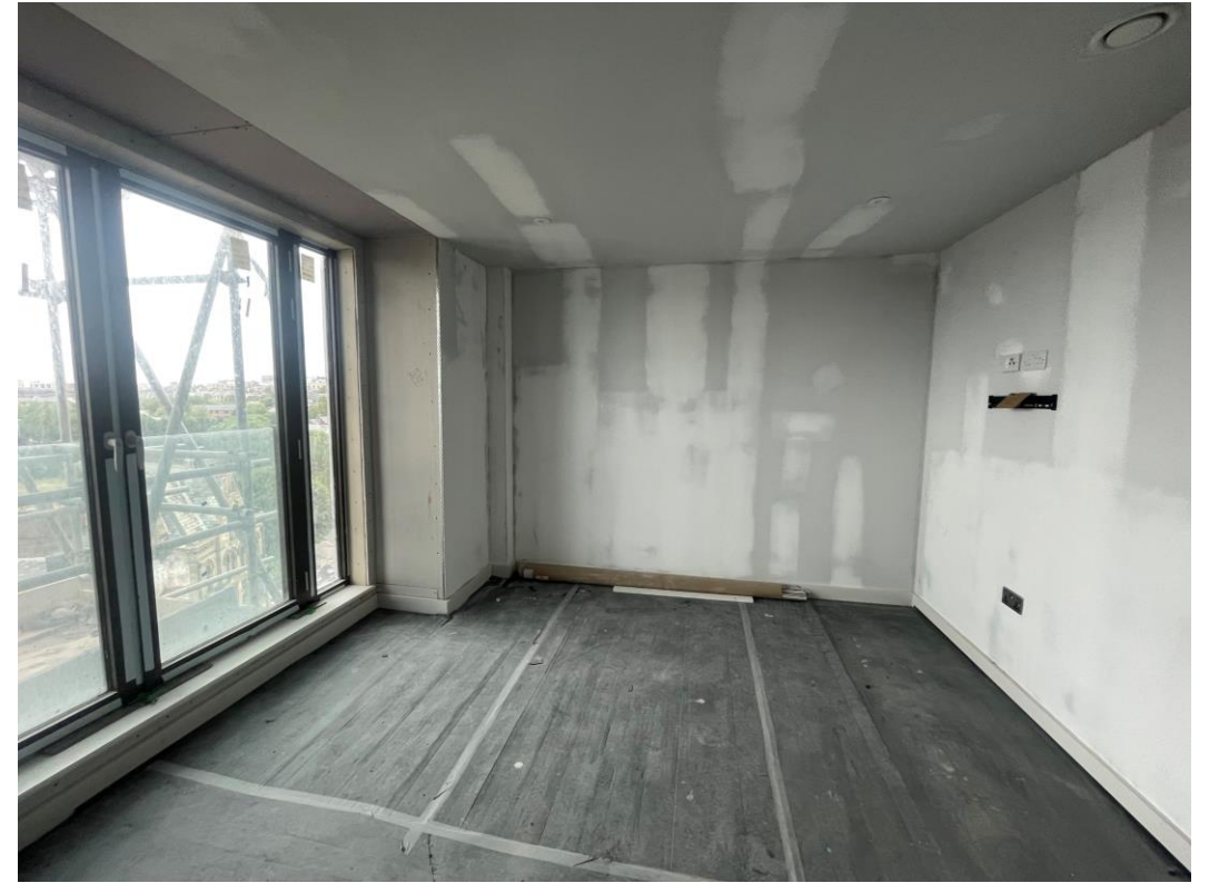
Laminate flooring installed and protected
