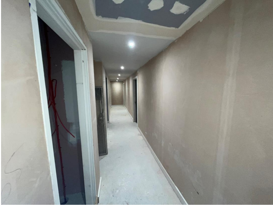
Circulation areas plastered
