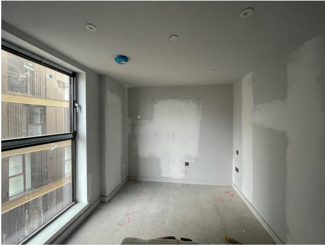
Bedroom finishes ongoing
