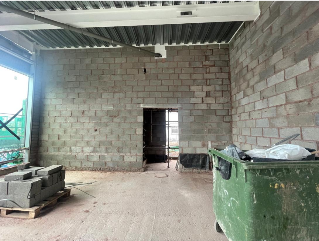
Masonry wall installed to Commercial Unit
