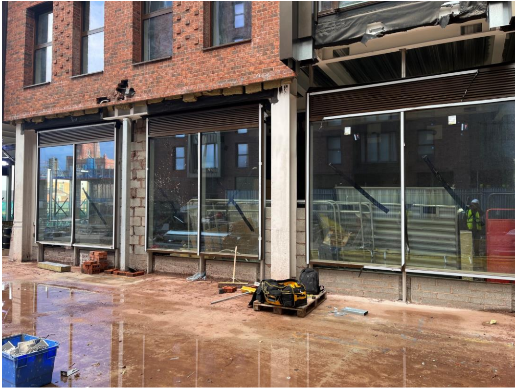
Block B – Curtain walling installation ongoing
