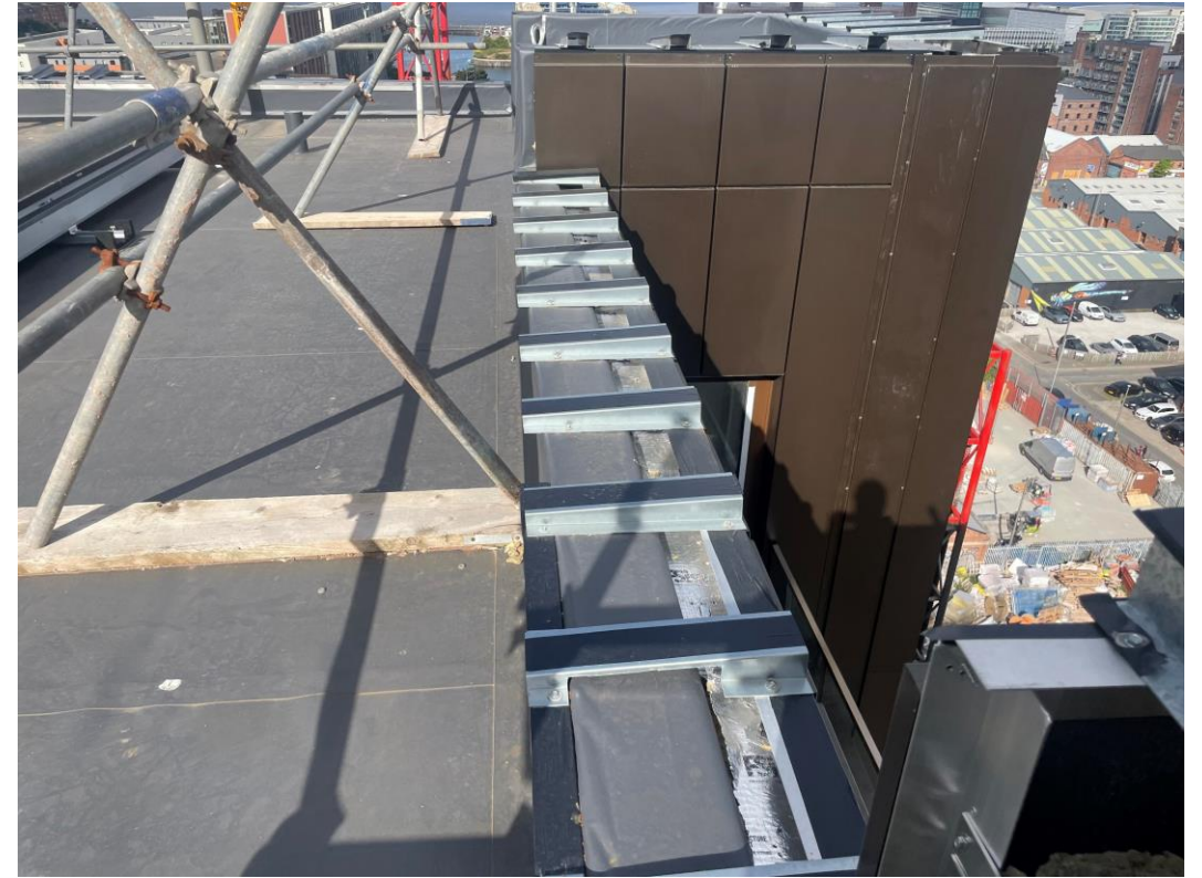
Cladding capping details installation ongoing
