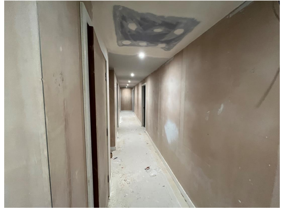
Circulation areas plastered
