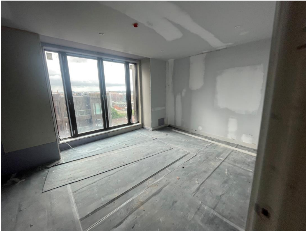
Lounge Finishes ongoing
