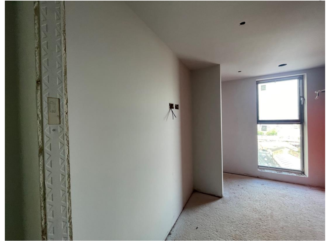
2 nd Coat decoration walls & ceilings
