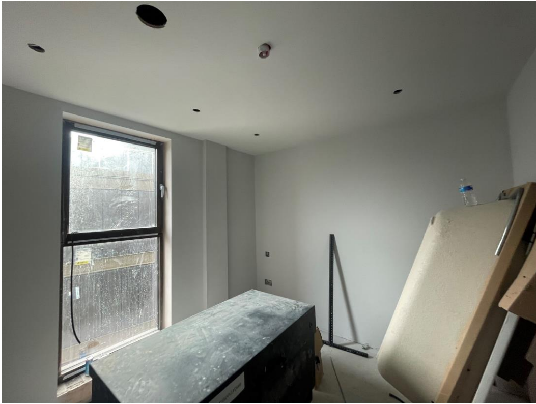
2 nd Coat decoration walls & ceilings
