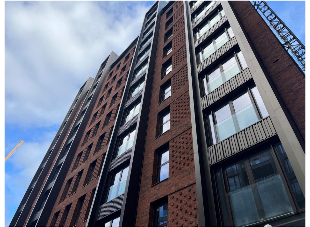
Block B – Brickwork & cladding installation
