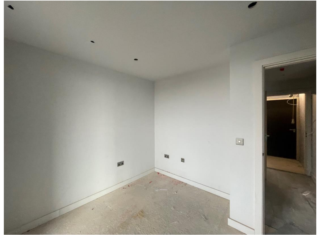
1st Coat decoration walls & ceilings
