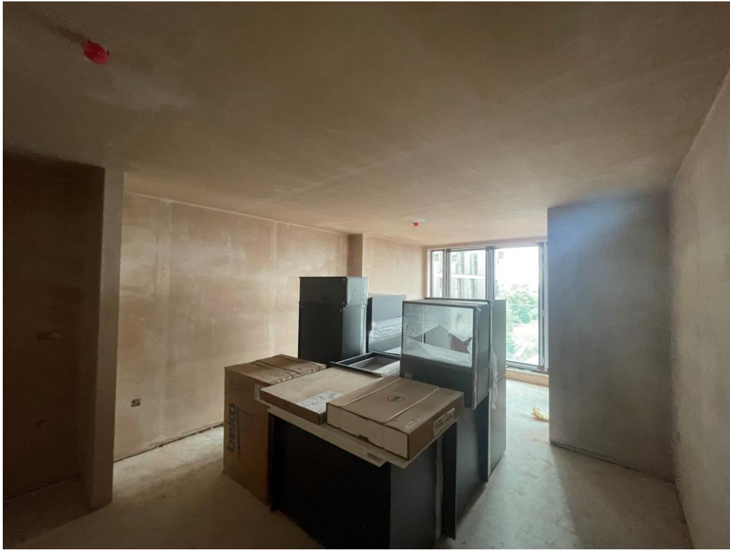
Kitchen / Lounge area walls & ceilings plastered
