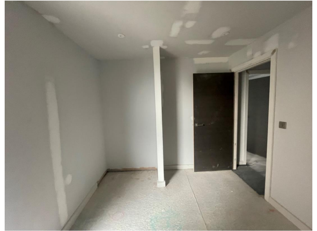
Bedroom finishes ongoing
