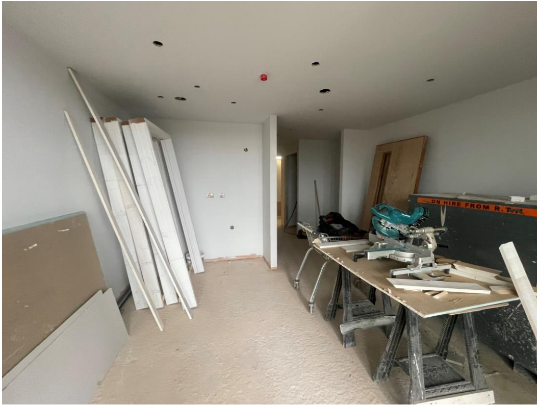
Hoist apartment fit-out
