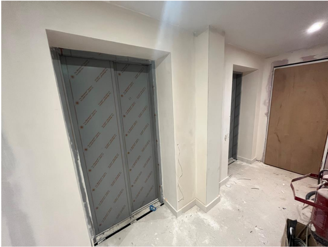
1 st coat decoration to walls & ceilings
