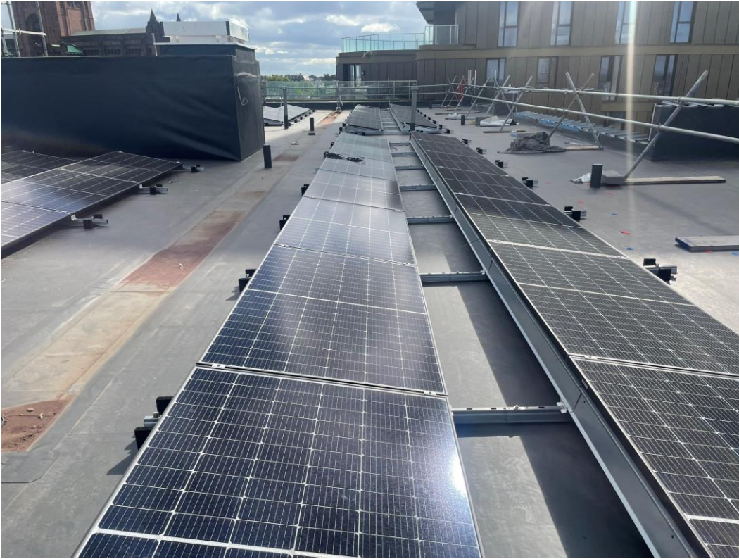
Solar panels installed
