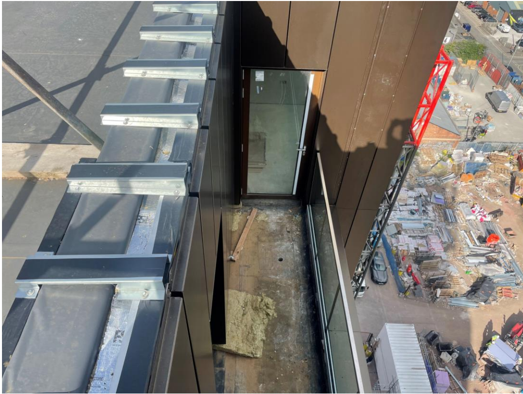
Cladding capping details installation ongoing
