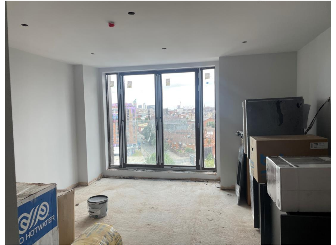
Lounge Finishes ongoing
