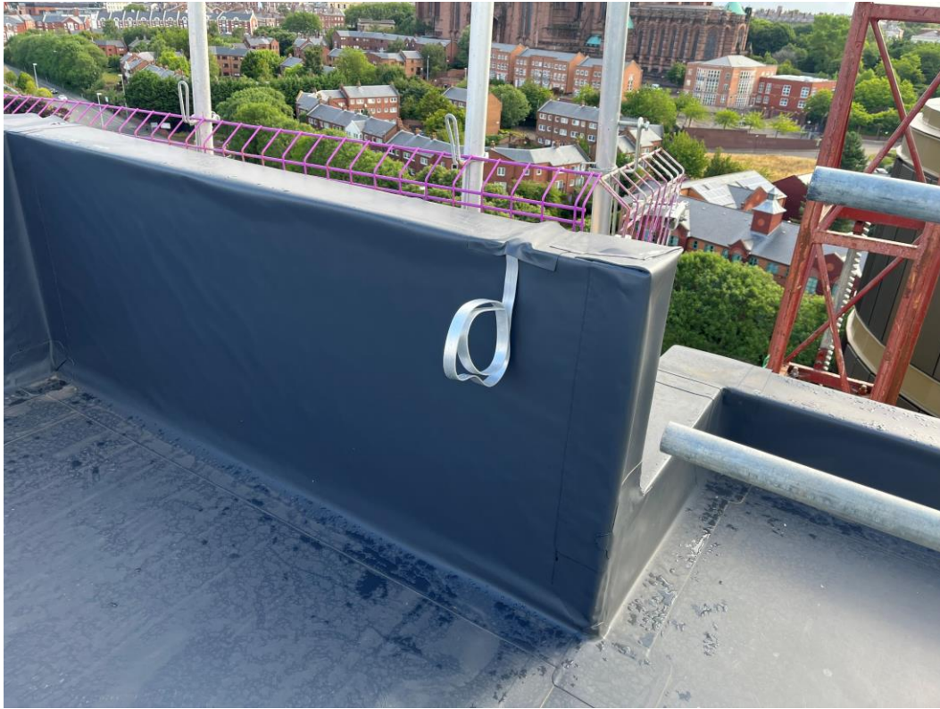
Roofing system installation complete
