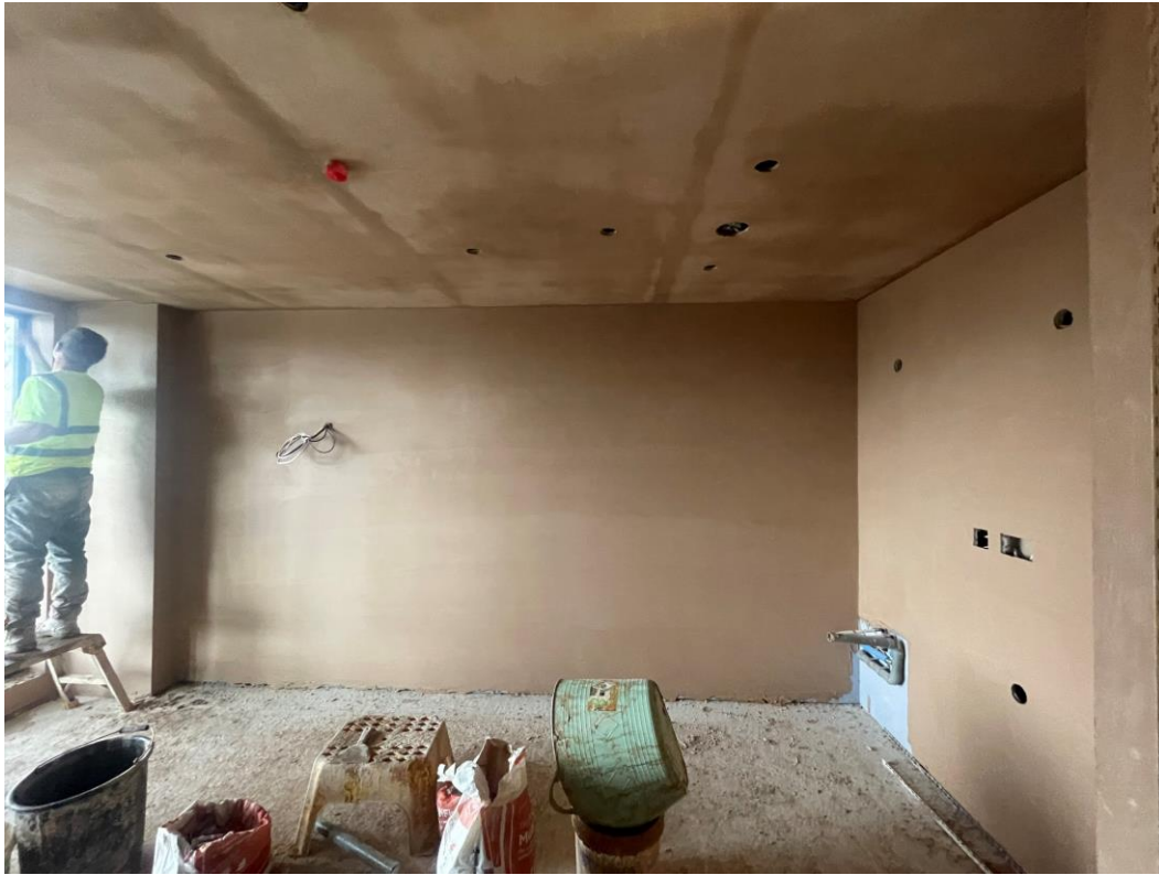
Apartment walls & ceilings plastered
