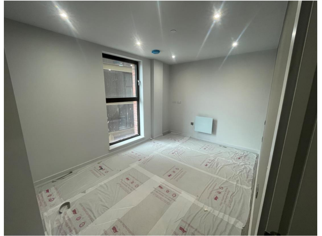
Bedroom carpets installed & protected
