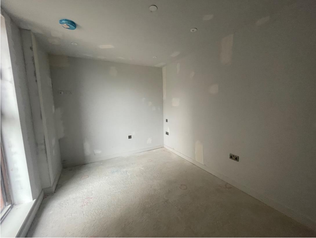
Bedroom finishes ongoing
