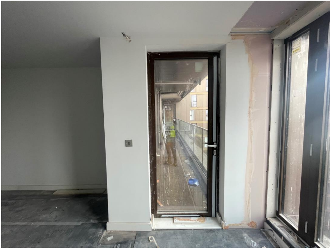
1st Coat decoration walls & ceilings
