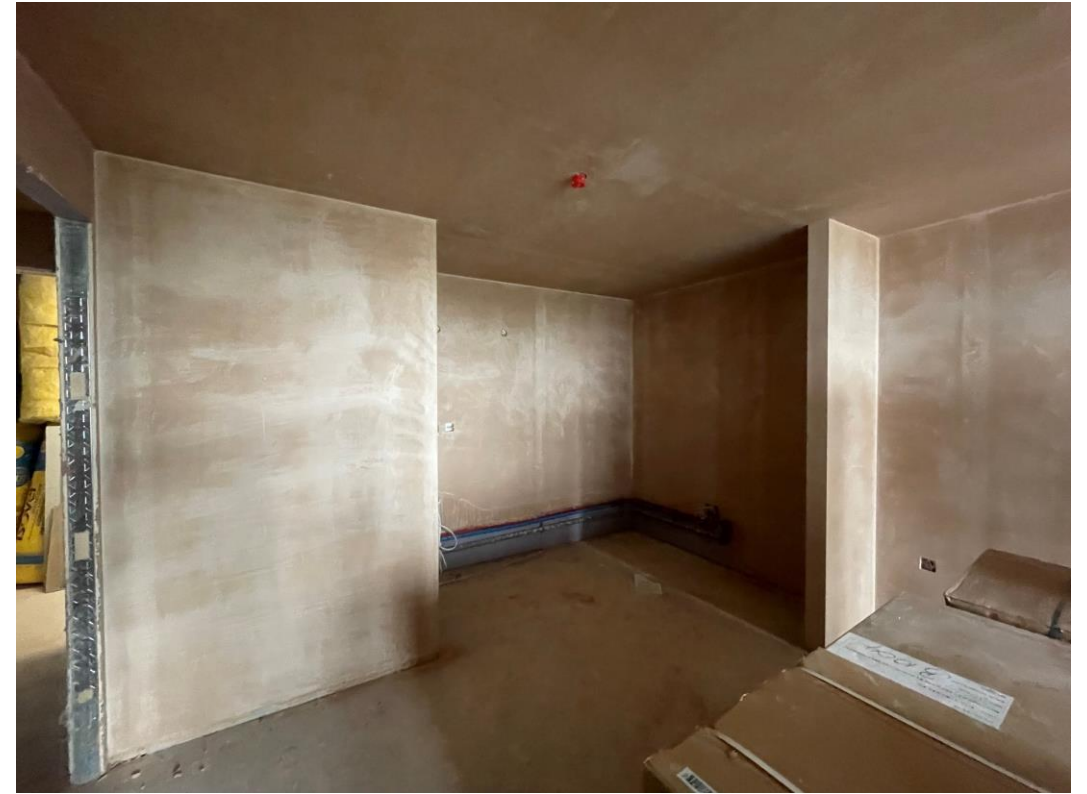
Kitchen / Lounge area walls & ceilings plastered
