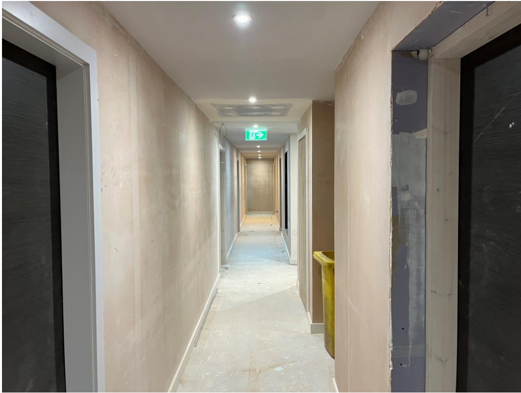
Circulation areas plastered
