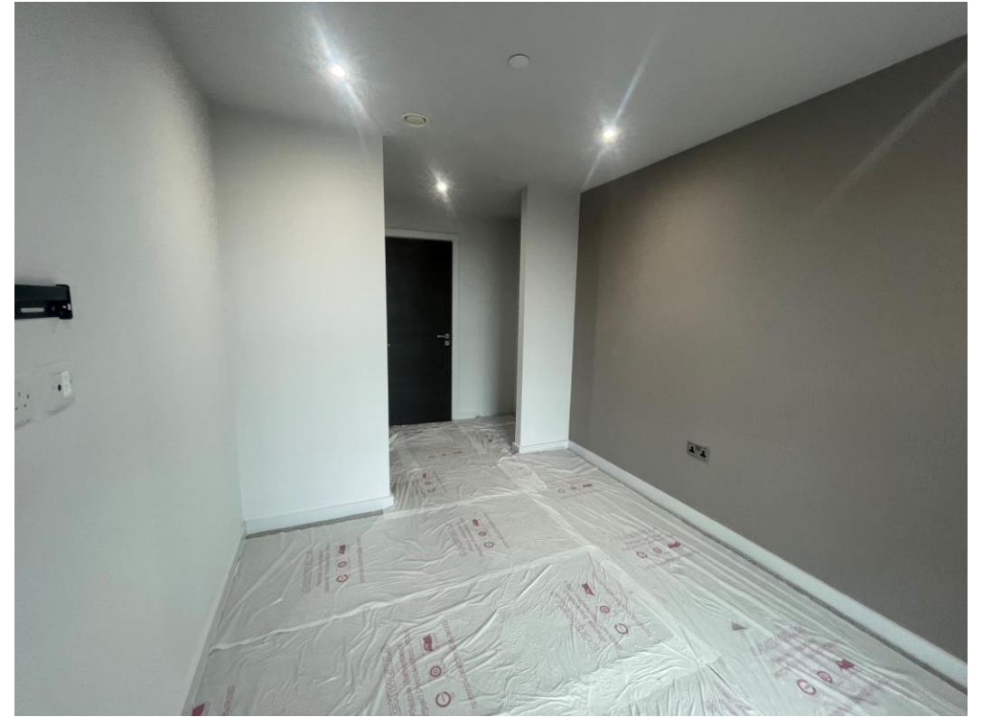
Bedroom carpets installed & protected
