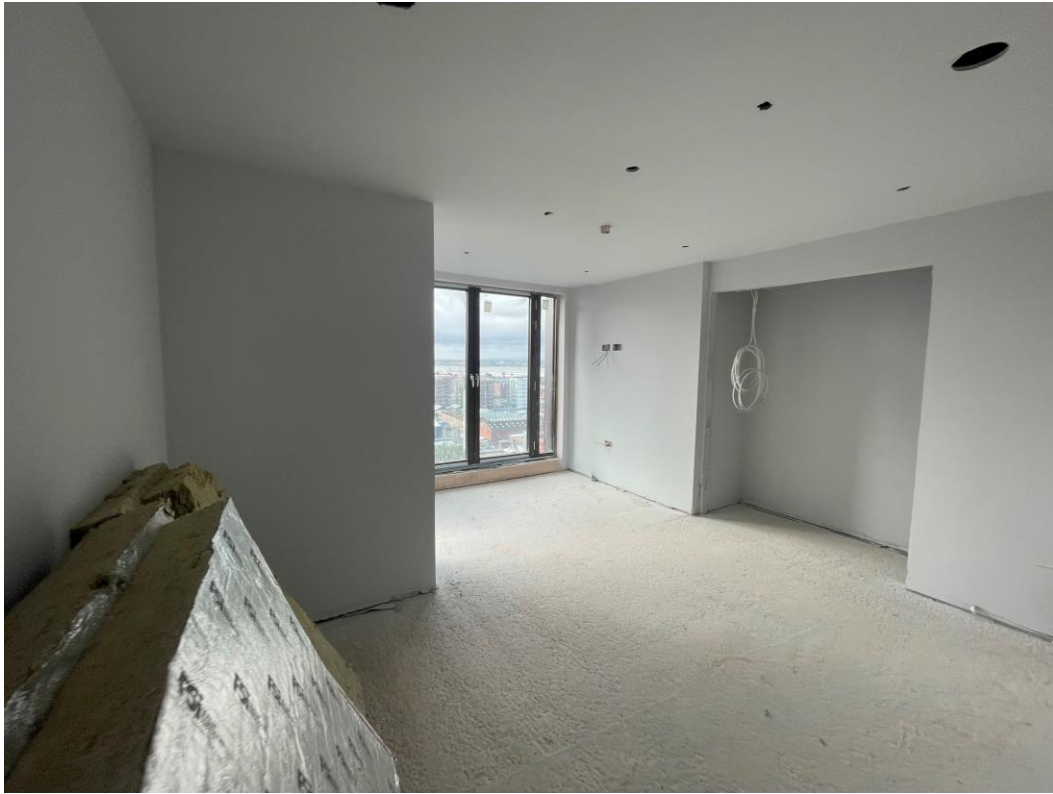
2 nd Coat decoration walls & ceilings
