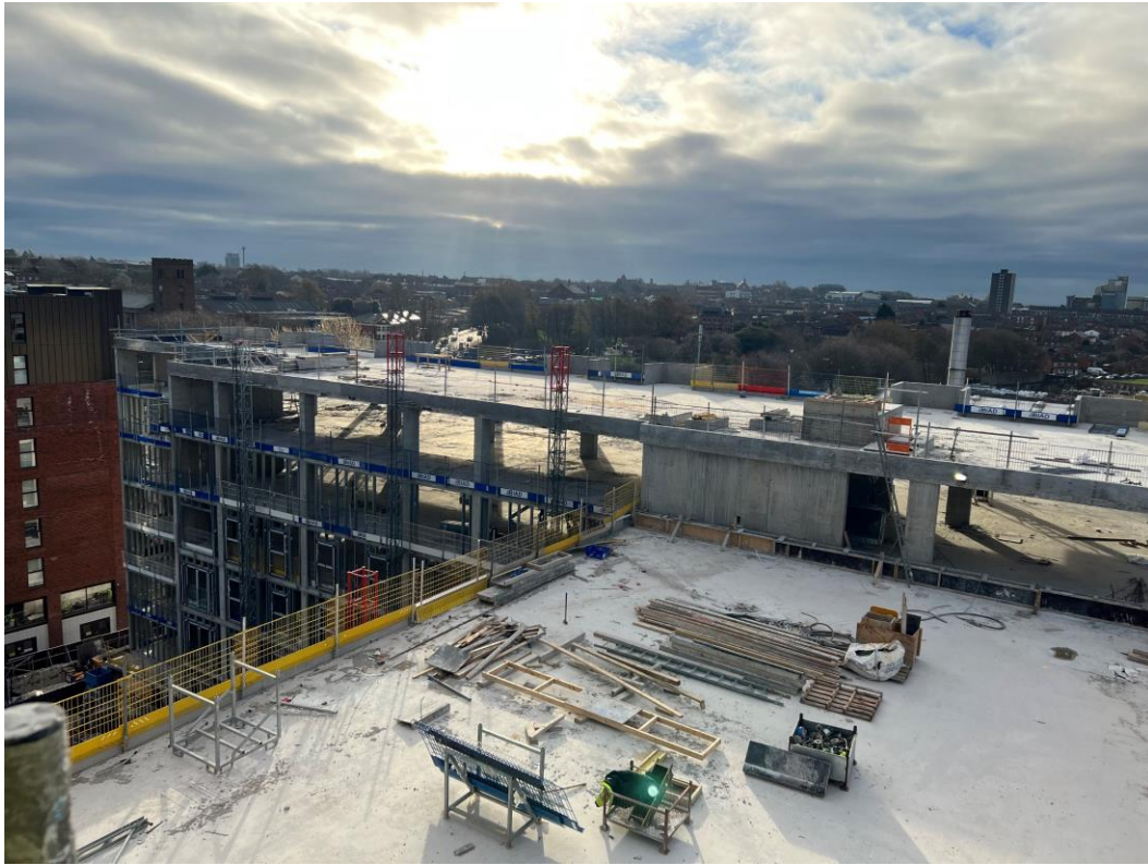
Block D Section B – Viewed from Section A
