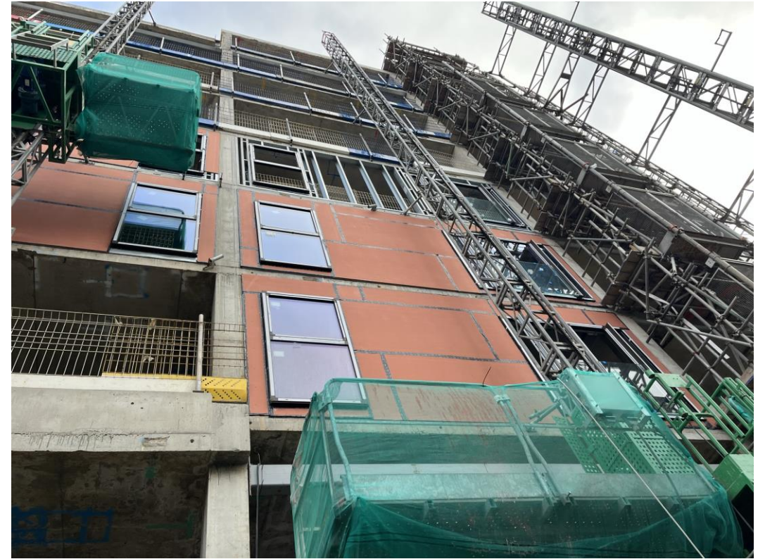
Block D Section B – Weatherboarding installation ongoing
