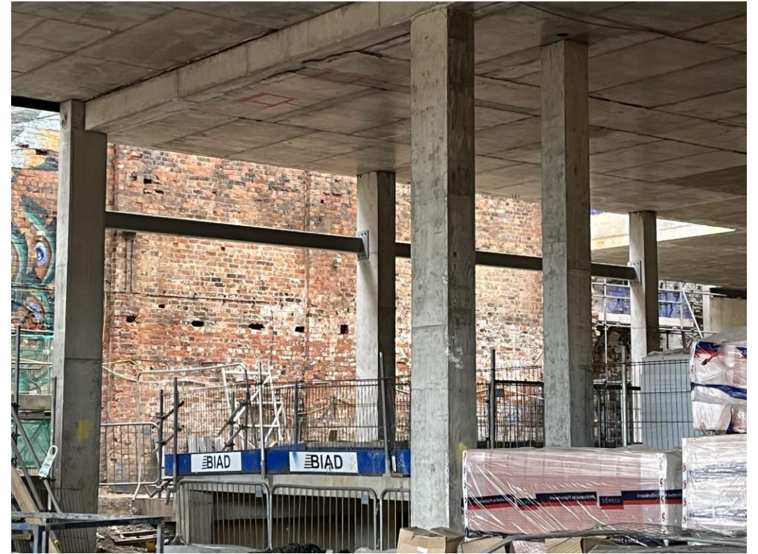
Structural support for curtain wall installation
