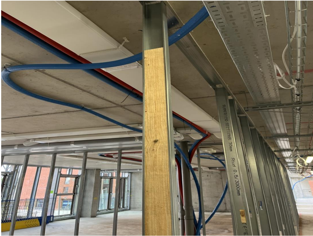
Pattress for doorframe installation
