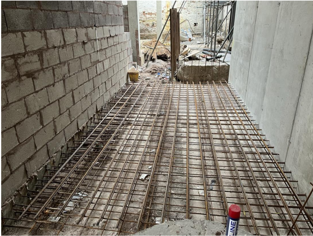
Ground Floor - Reinforcement in place for concrete slab pour
