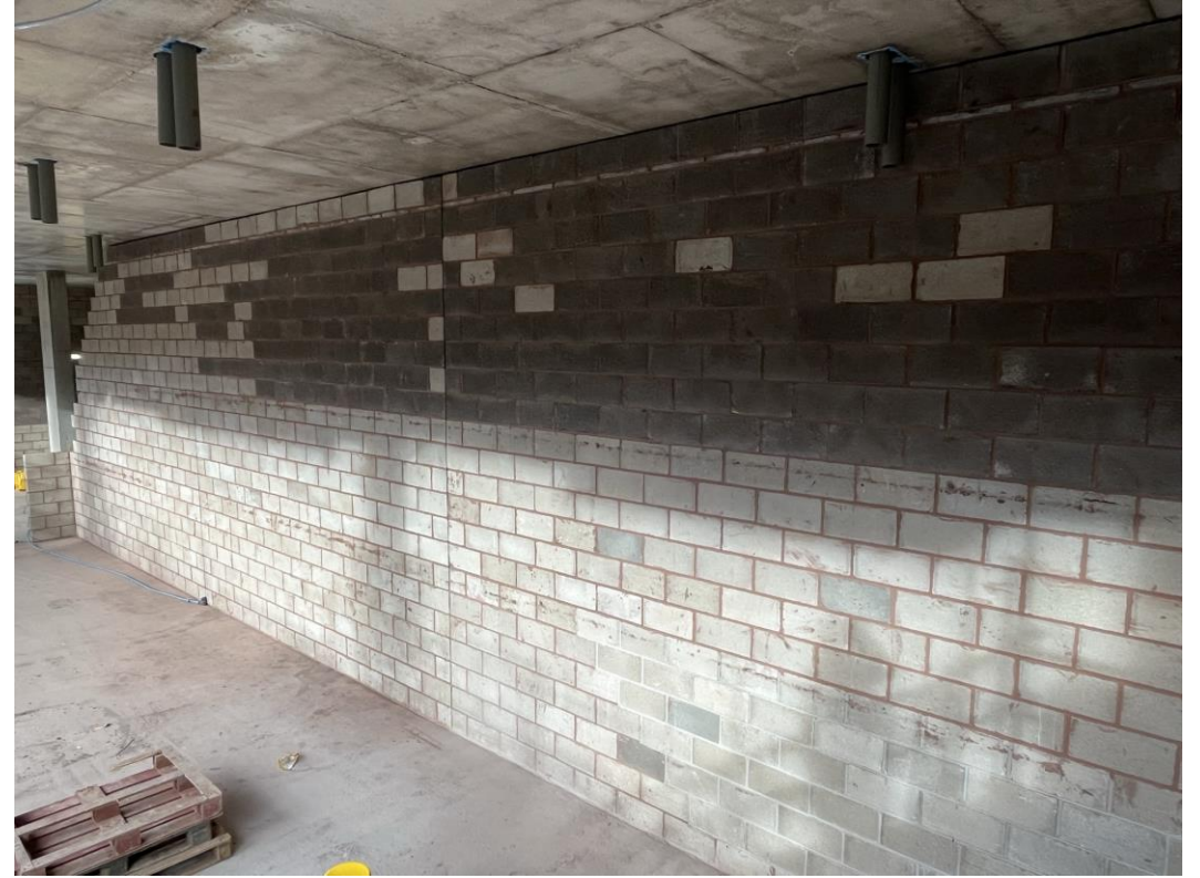
Ground floor blockwork walls
