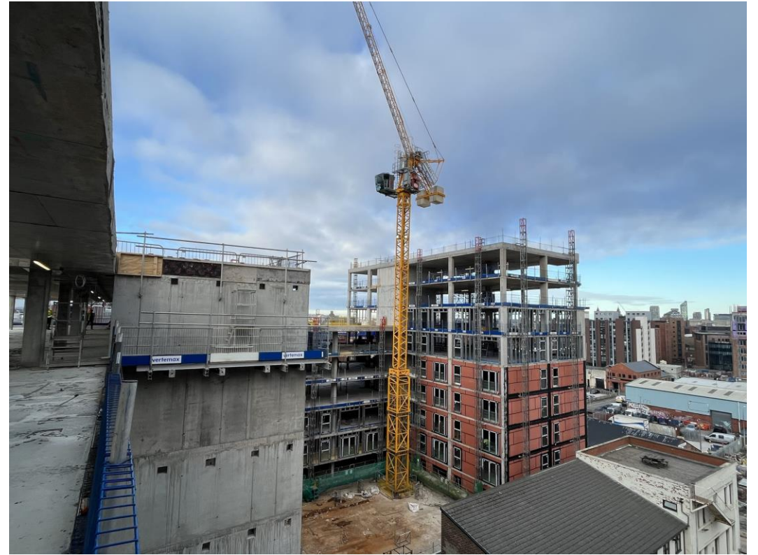
Block D Section A & C – Viewed from Section B
