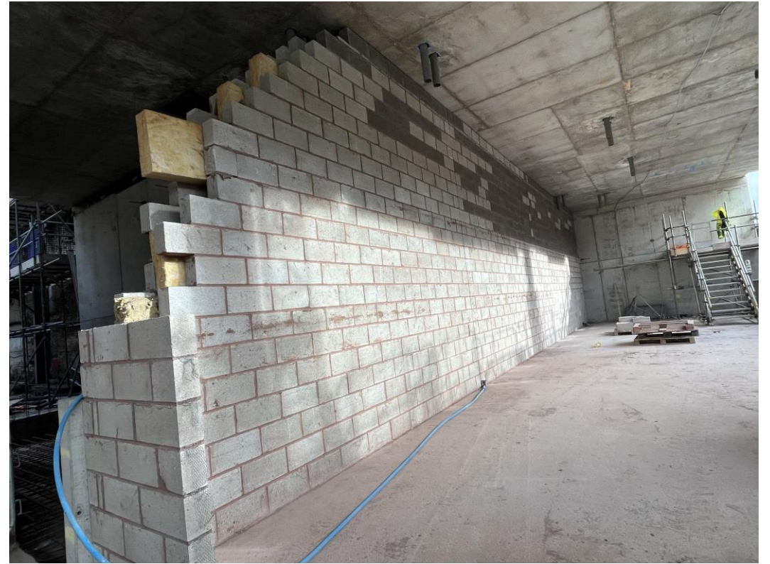
Ground floor blockwork walls
