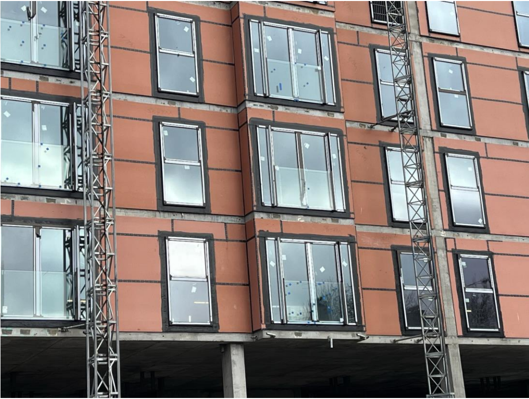
Block D Section B – Glazed units installed
