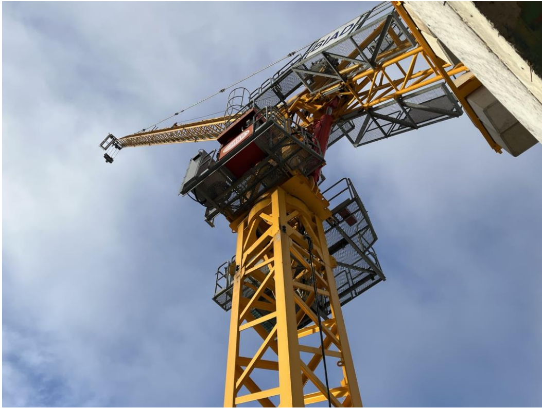
Block D – Crane in operation
