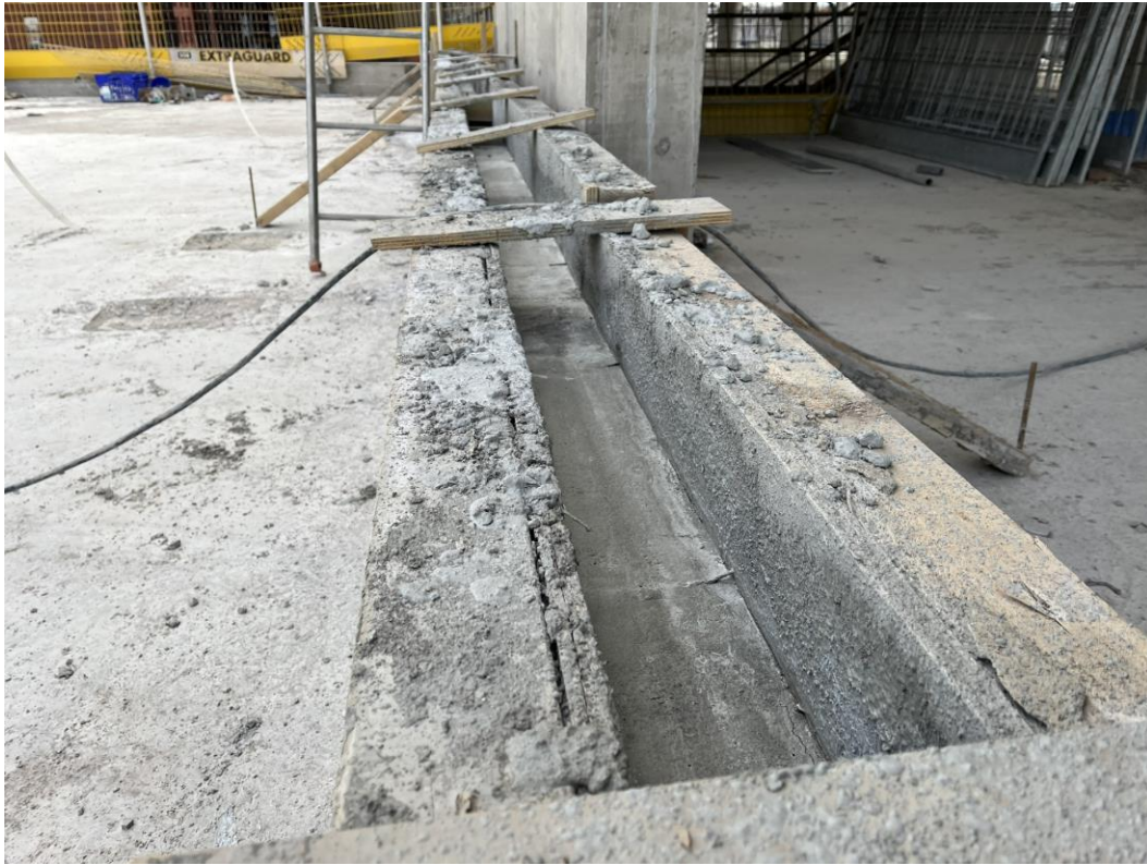
Block D Section B – Formation of concrete upstand
