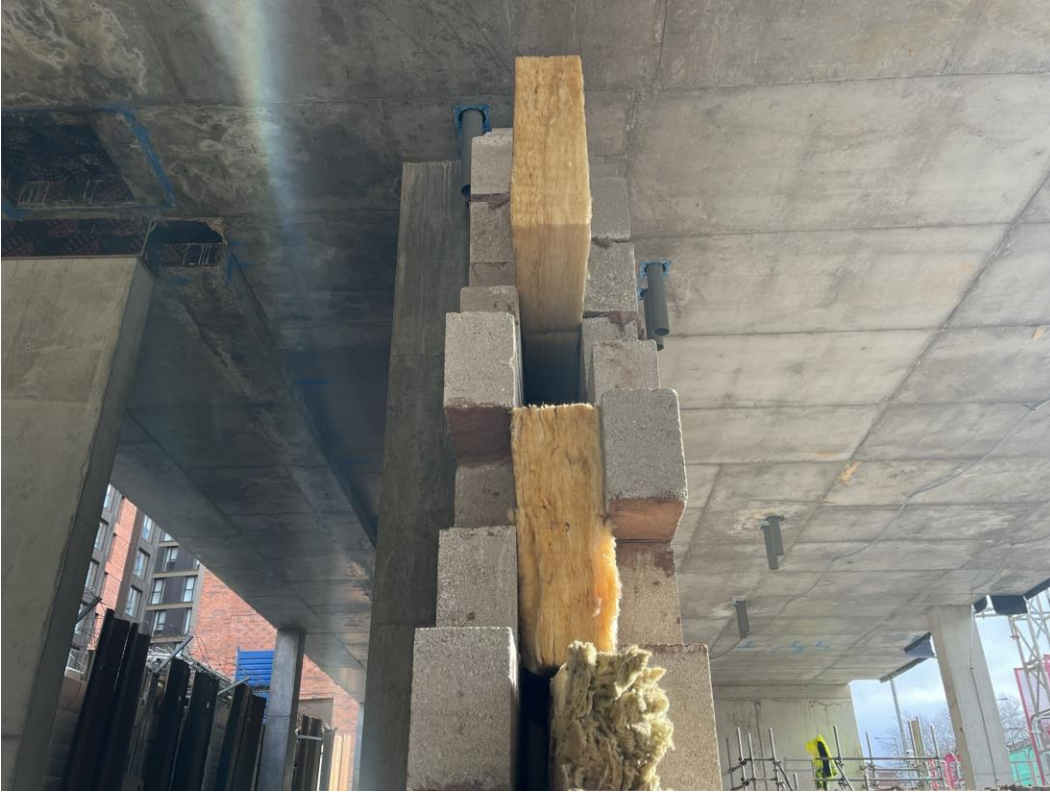
Cavity wall insulation
