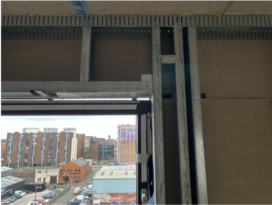
Interface between window and SFS
