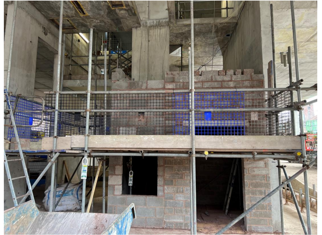
Ground floor blockwork walls
