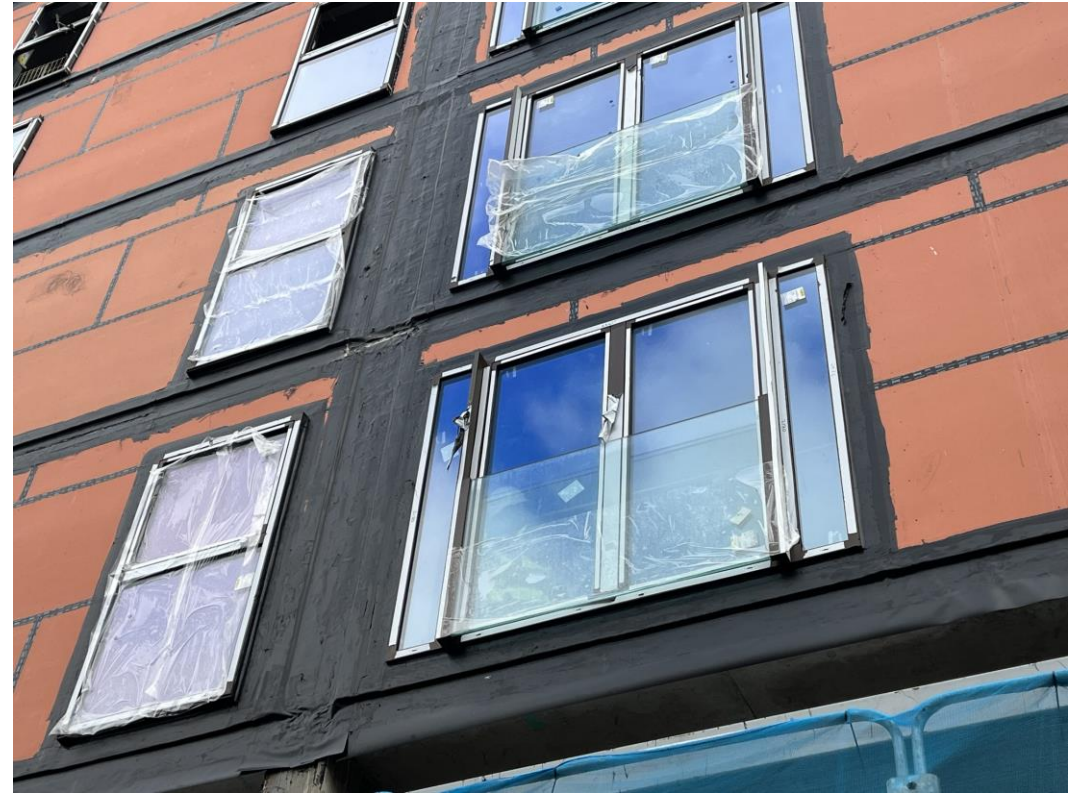
Block D Section B – Glazed balustrade installation ongoing
