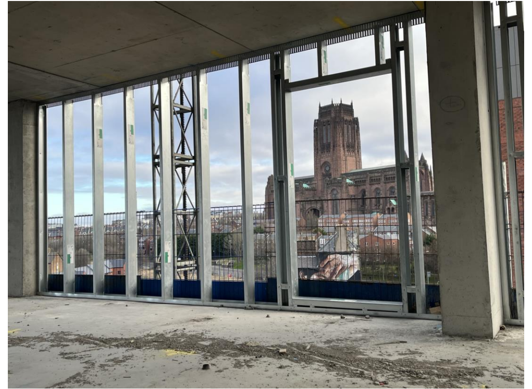
SFS Installation nearing completion
