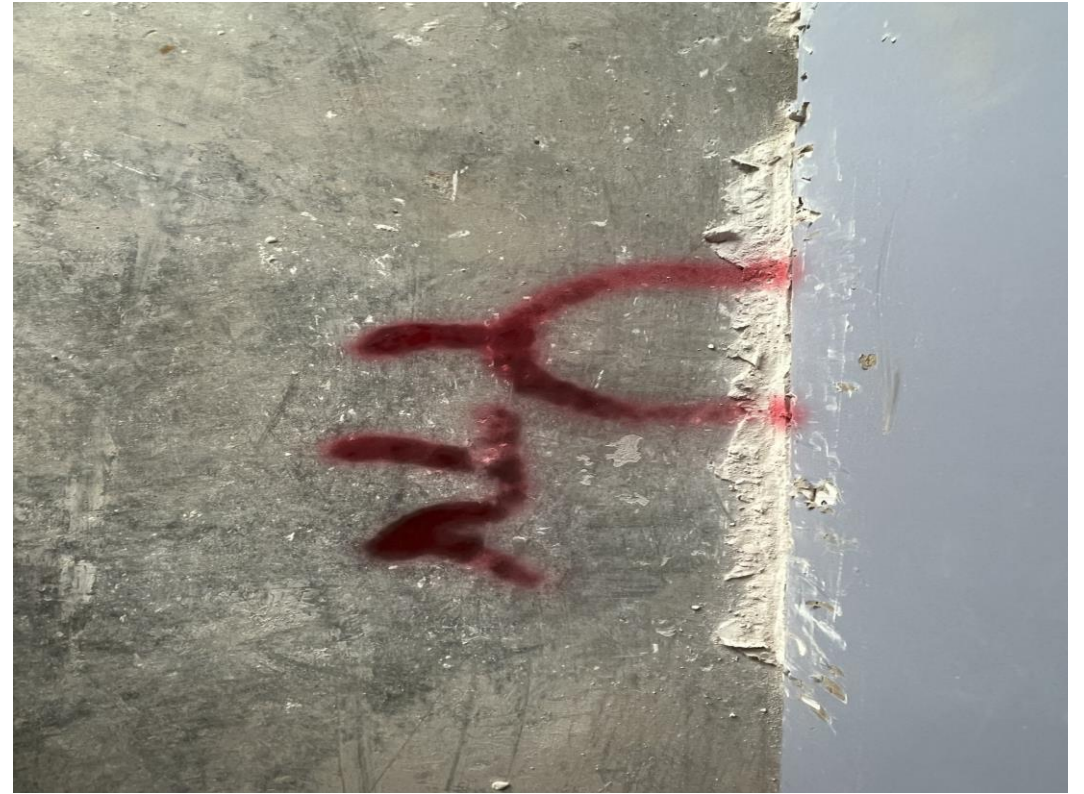
Setting out of first second electrical underpass
