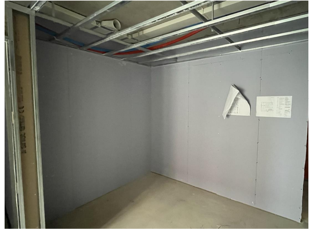
First side partition boarding commenced
