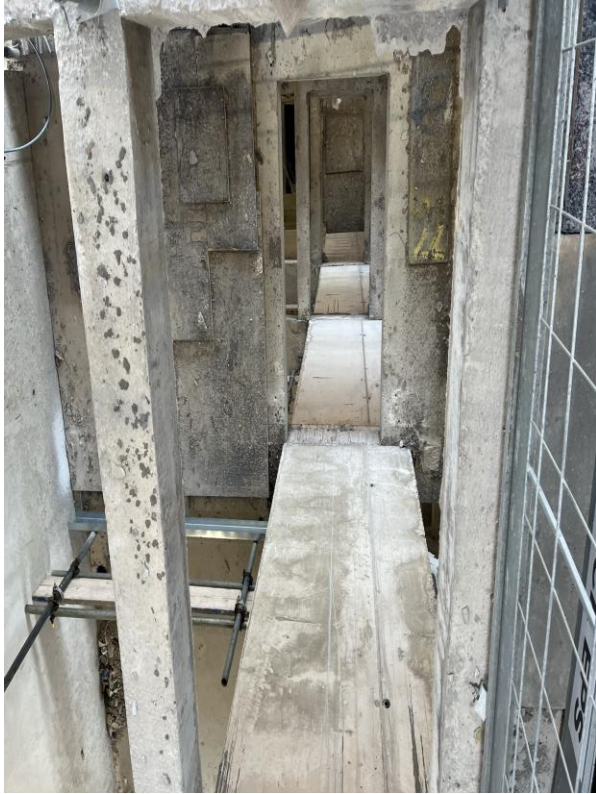
Openings for lift shaft
