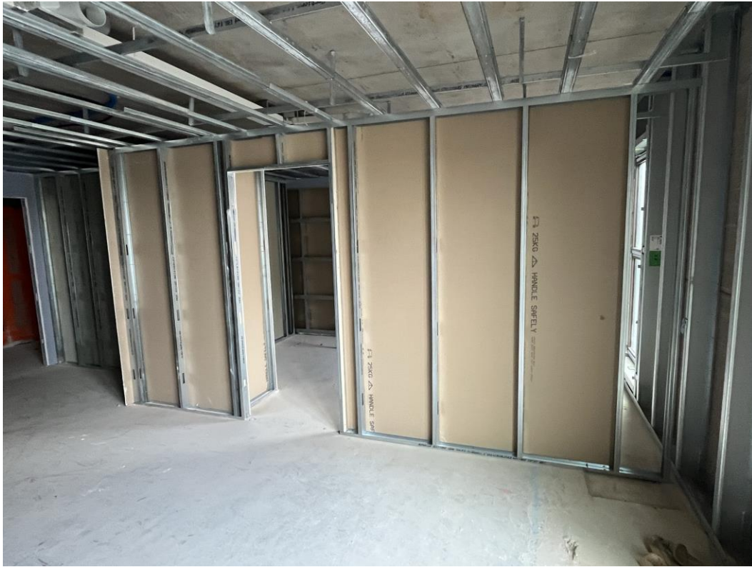
First side partition boarding commenced
