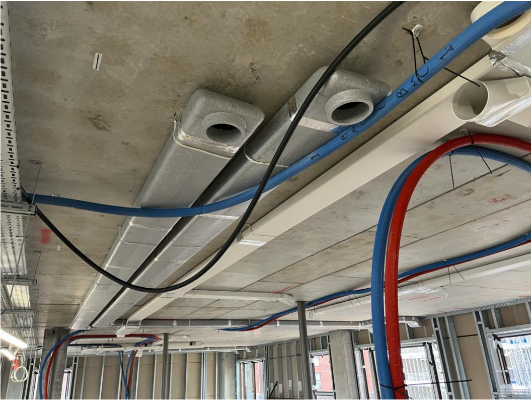
Block D Section A – Mechanical ductwork installed
