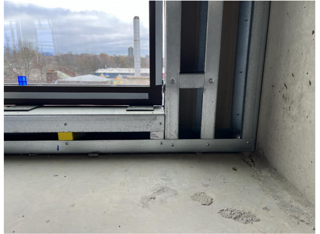
Interface between window and SFS
