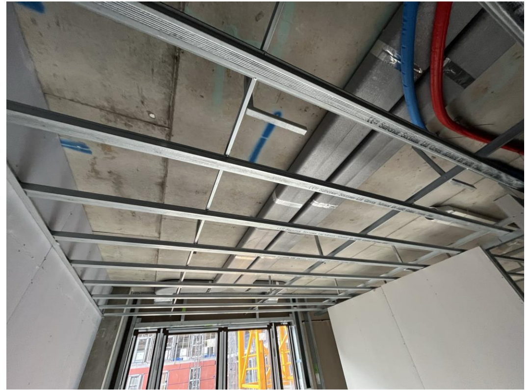
Suspended ceiling installation commenced
