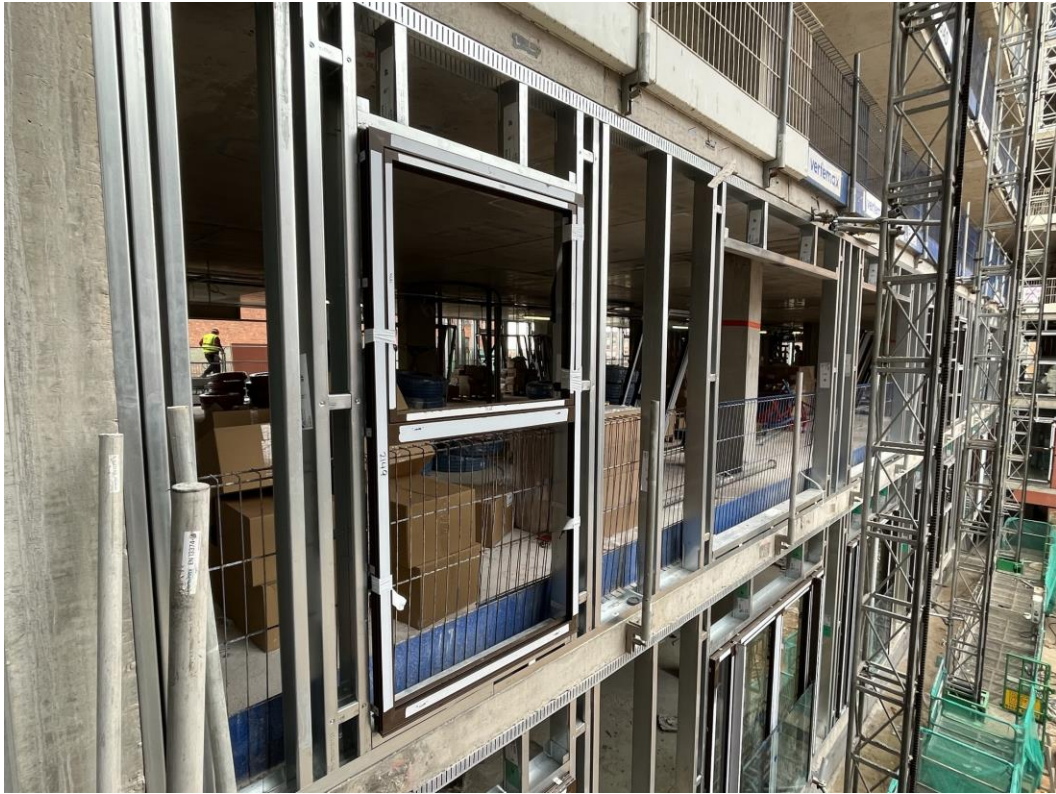
External windows installed
