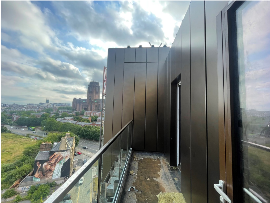
Cladding installation
