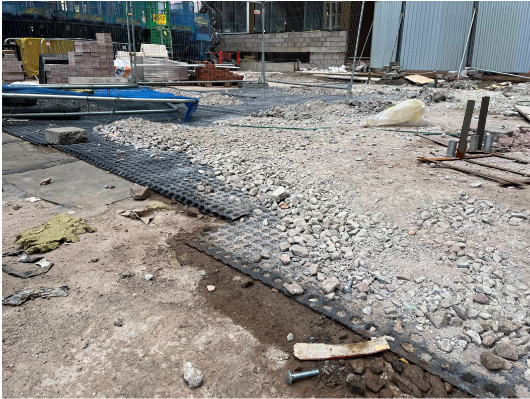
Podium build-up installation
