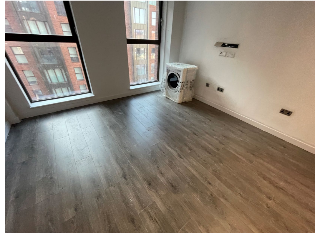
Laminate installed
