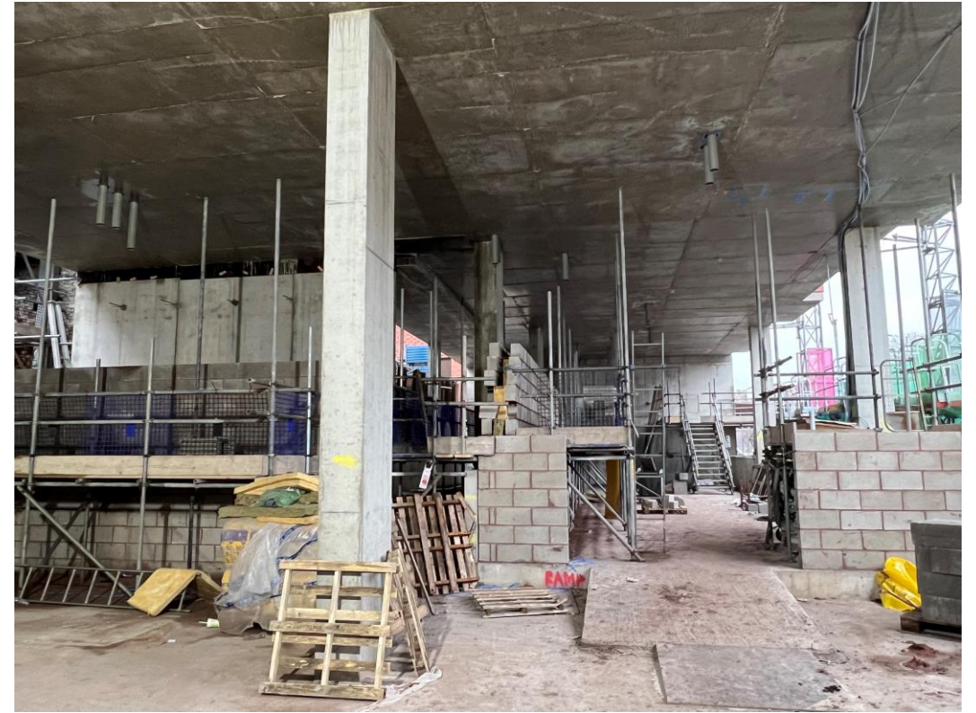
Ground Floor blockwork ongoing
