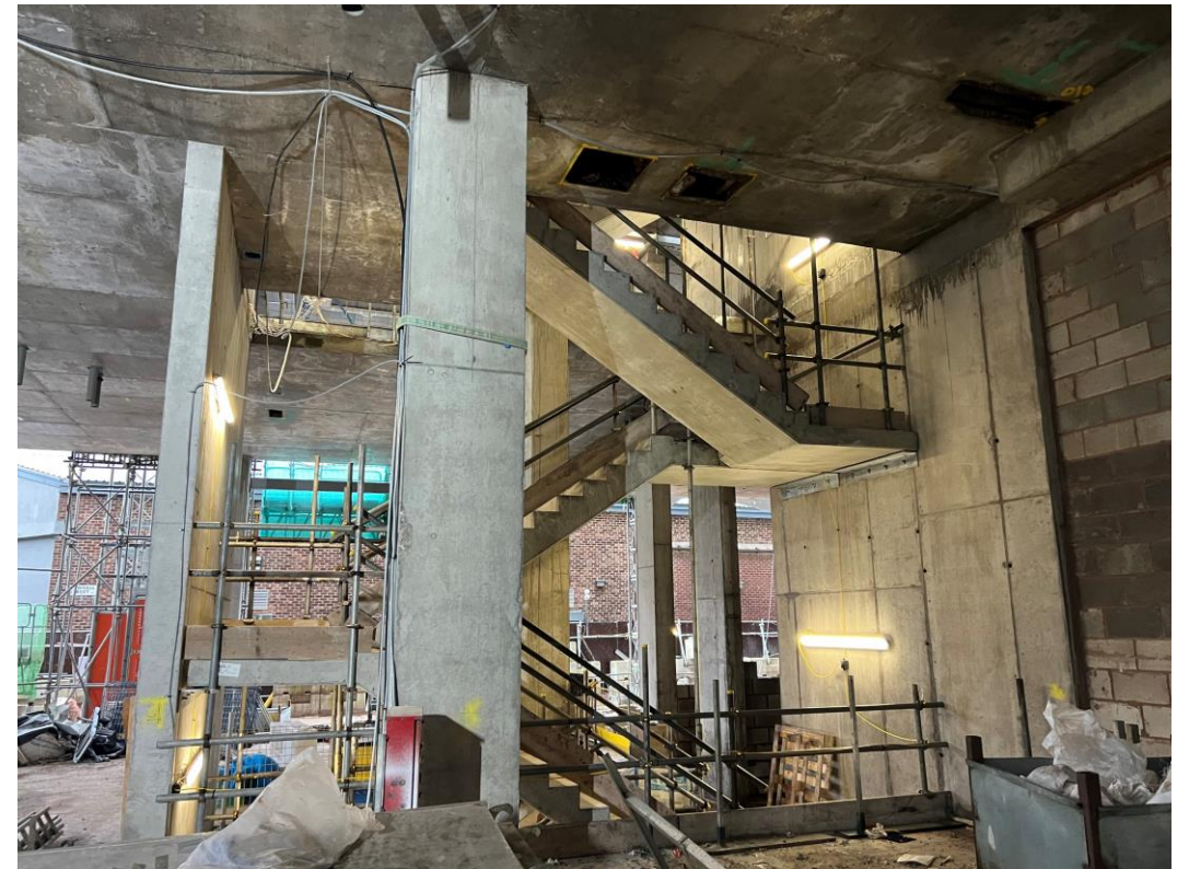
Block D Section B – Pre-cast concrete staircase
