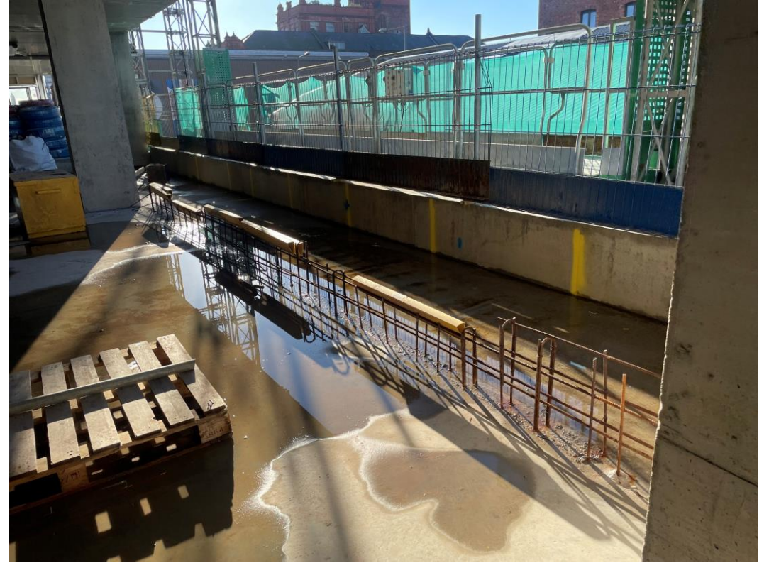
Reinforcement in place for formation of concrete upstand
