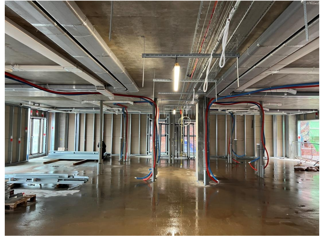
Block D Section A – Mechanical ductwork installed
