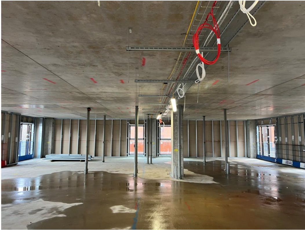
Electrical containment installation ongoing
