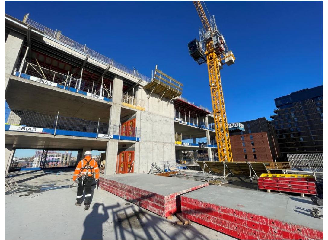
Block D Section A – Viewed from Section C
