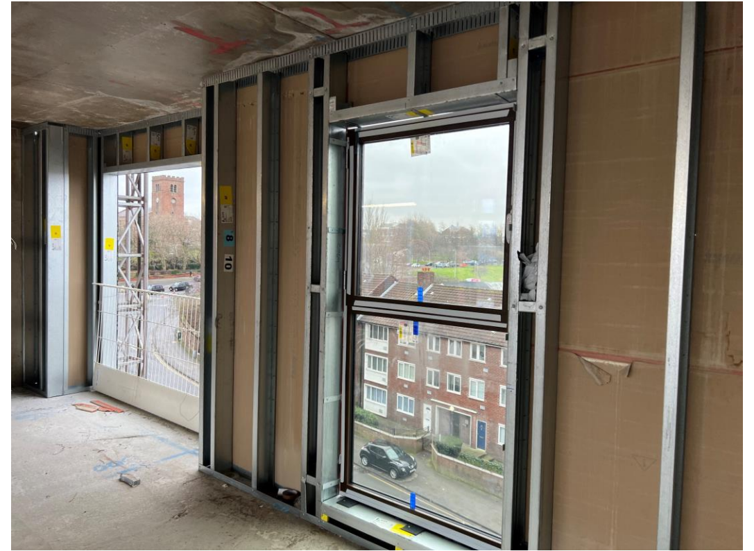
External windows installed
