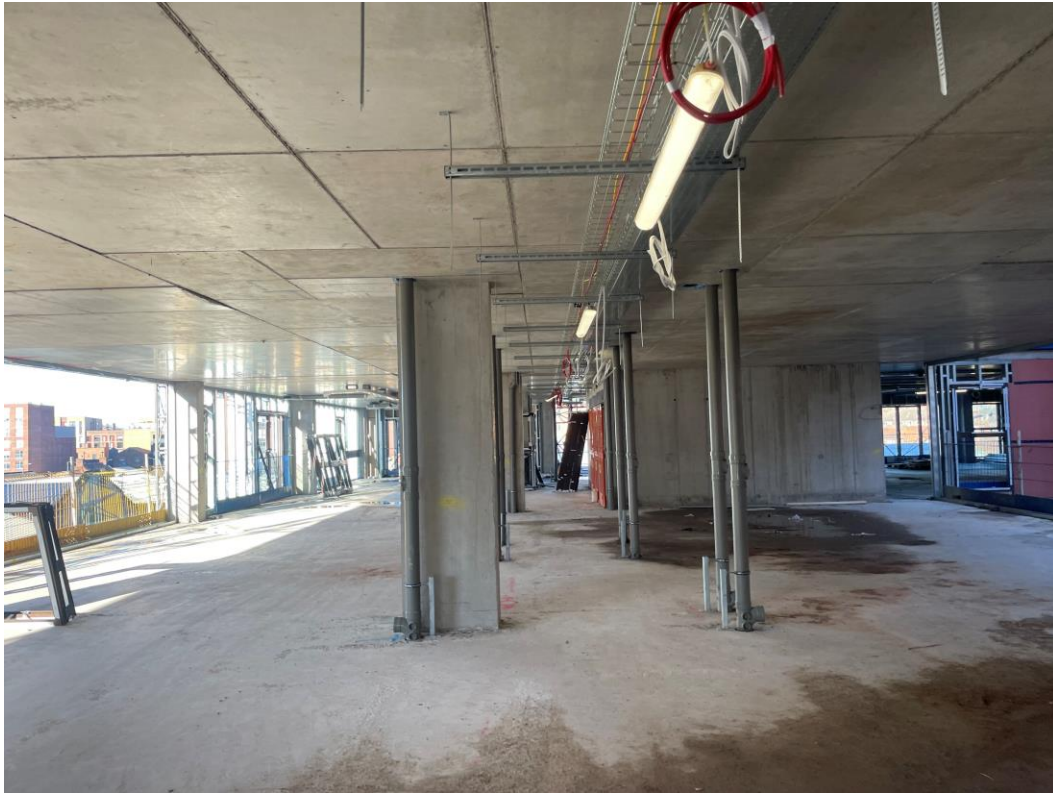
Electrical containment installation ongoing
