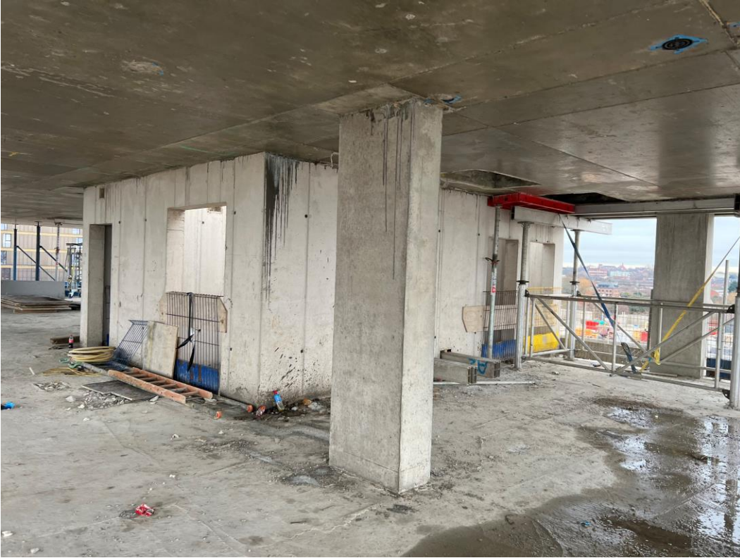
Concrete frame structure complete
