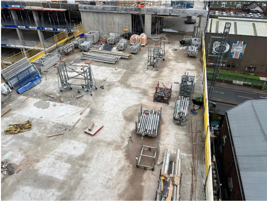
Block D Section C – Viewed from Section A
