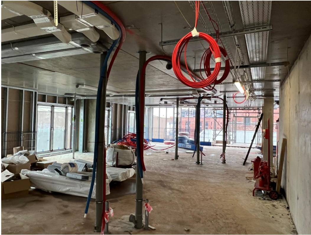
1 st Fix M&E commenced to lower floor levels
