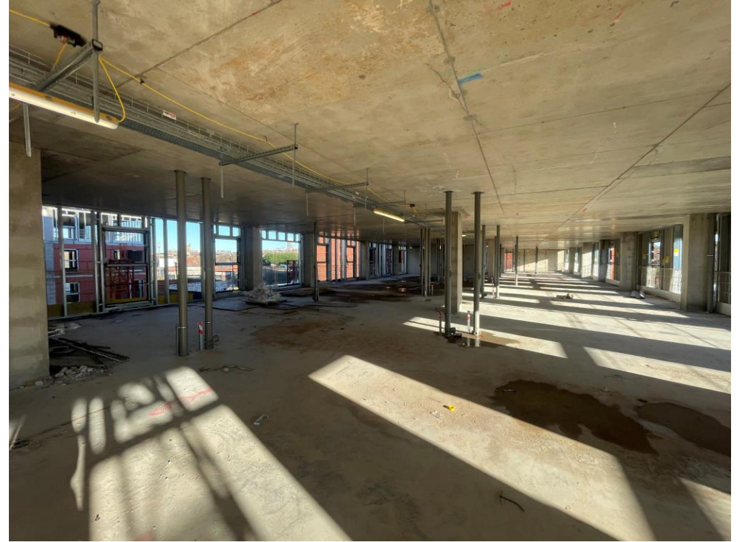
Electrical containment installation ongoing
