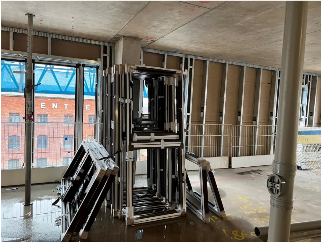
External windows onsite
