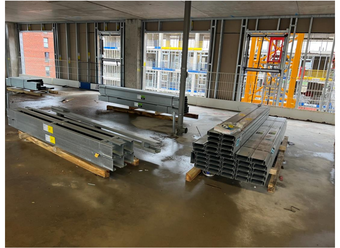
SFS loaded for installation
