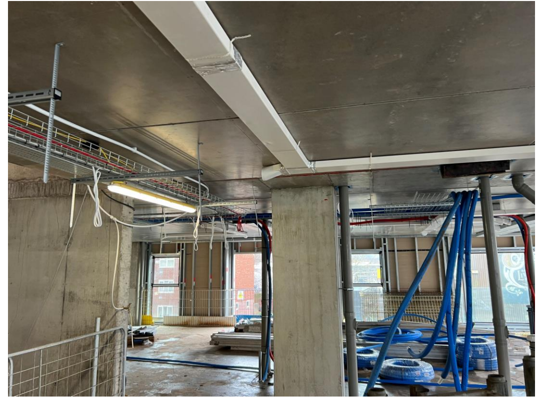
Block D Section A – Mechanical ductwork installed
