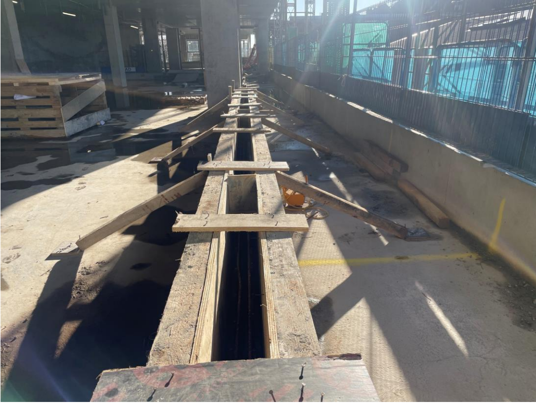
Formwork in place for casting of concrete upstand
