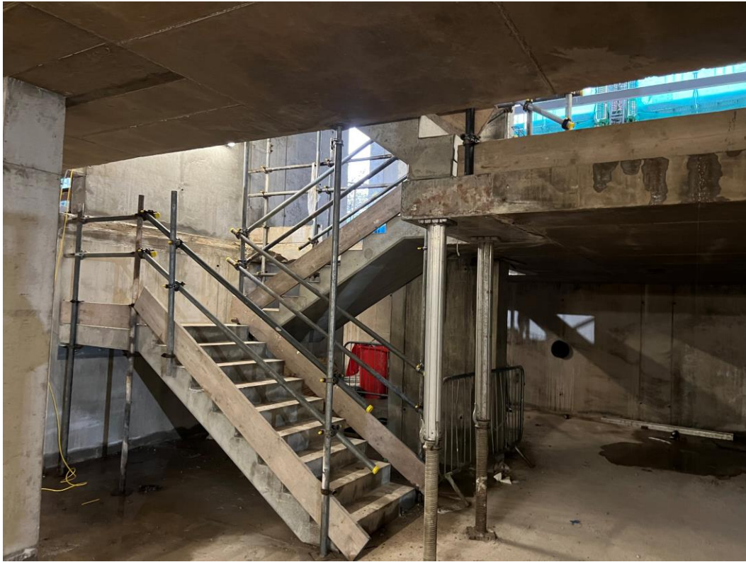
Block D Section B – Pre-cast concrete staircase
