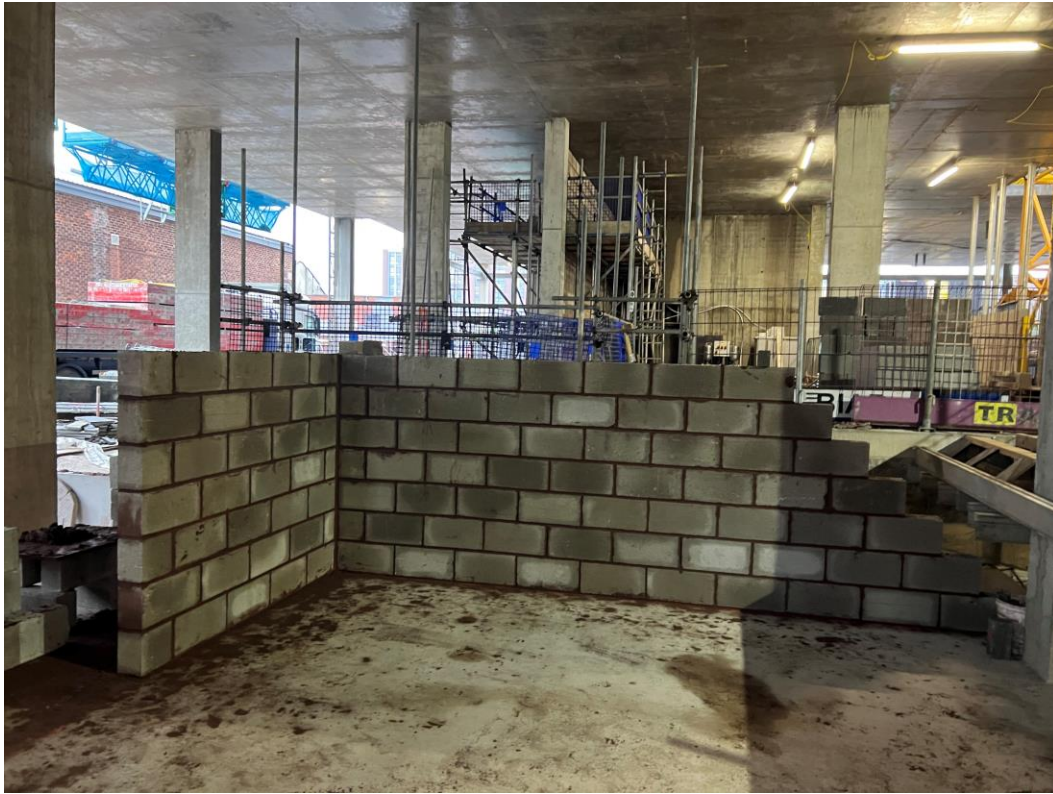
Ground floor blockwork walls
