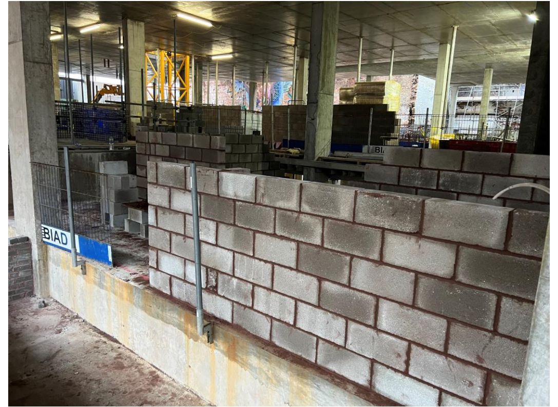
Ground floor blockwork walls
