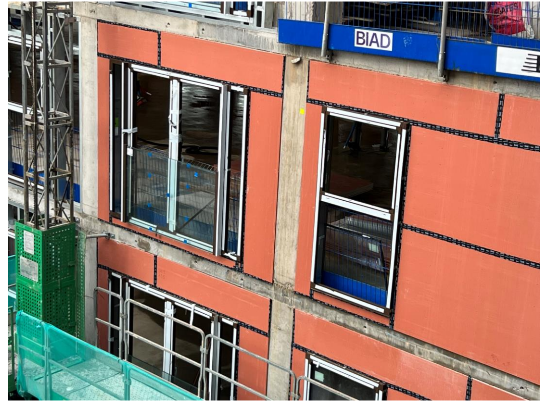
Window & weatherboarding installation ongoing
