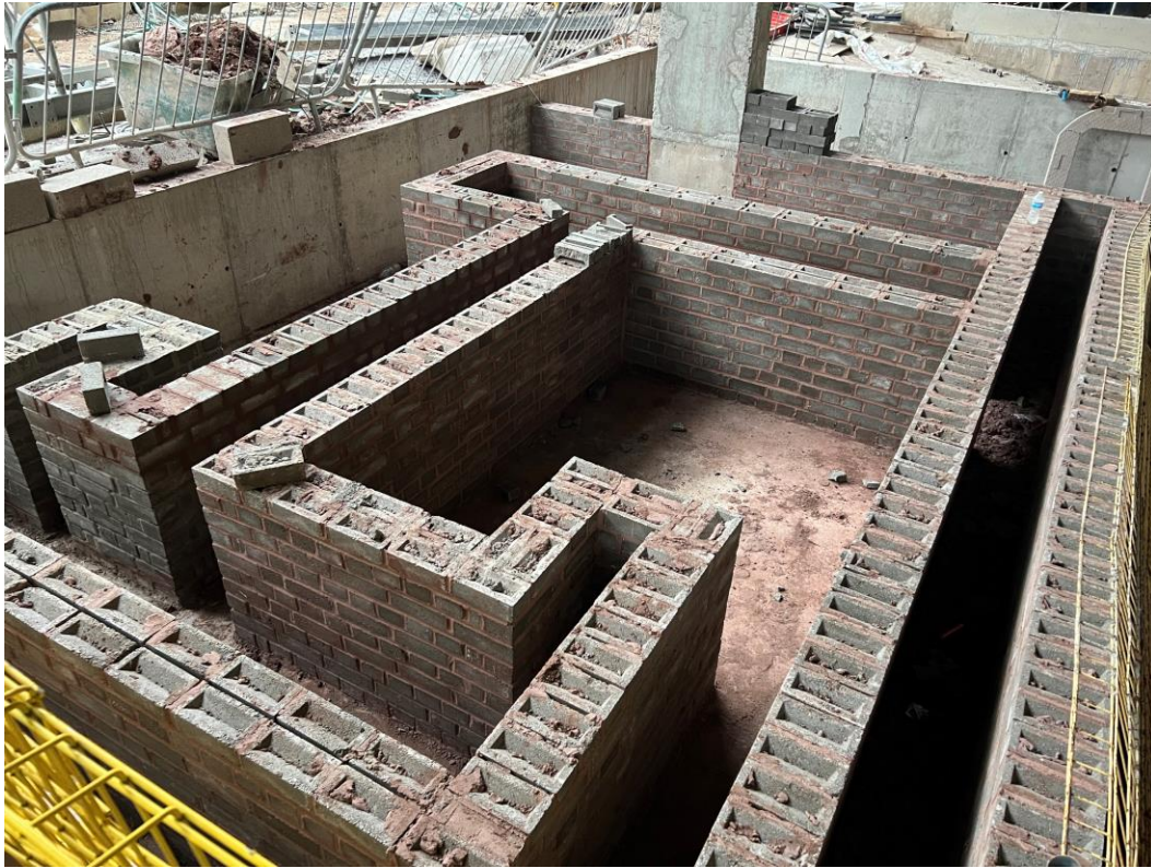
Ground floor blockwork walls
