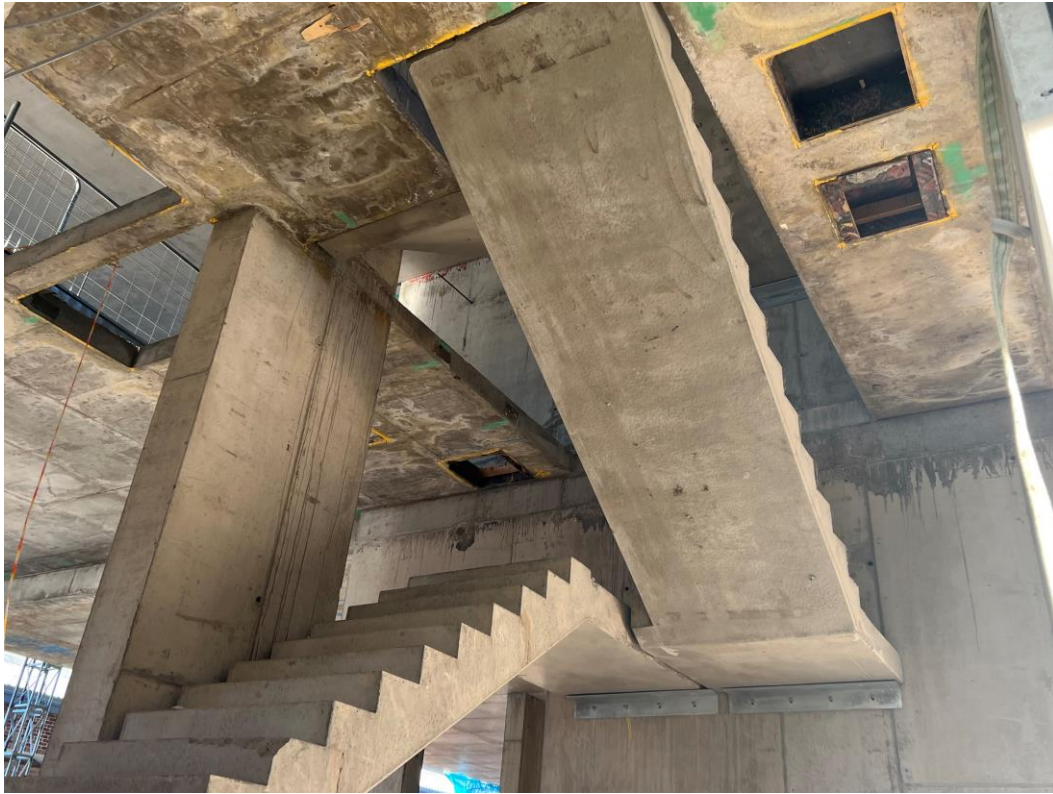
Block D Section B - Pre-cast concrete staircase
