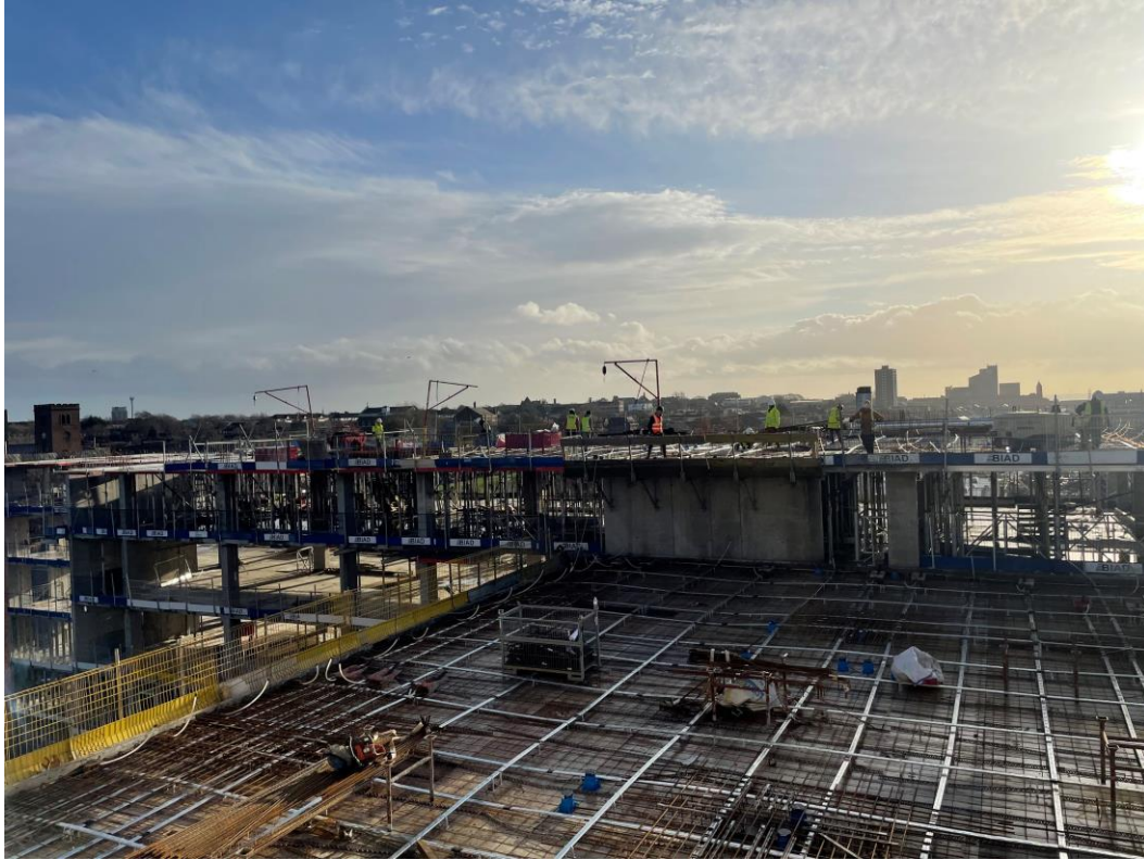
Block D Section B – Reinforcement in place for concrete slab pour
