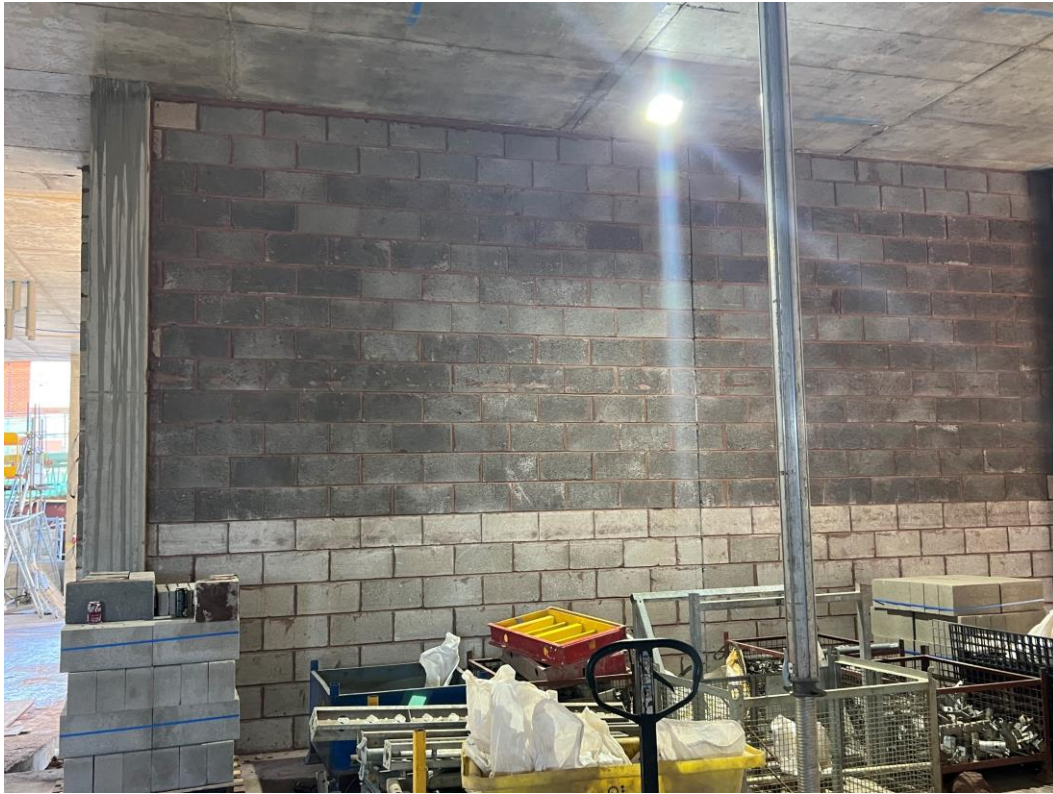
Ground floor masonry walls
