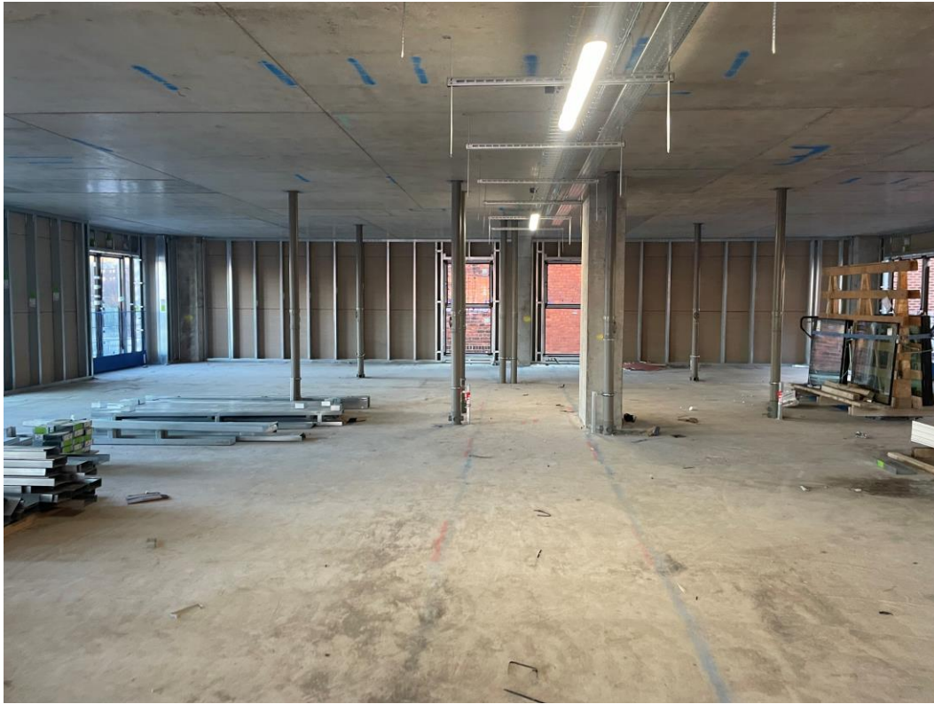
Electrical containment installed has commenced
