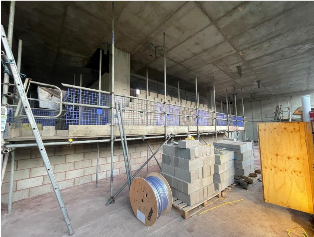
Ground floor masonry walls
