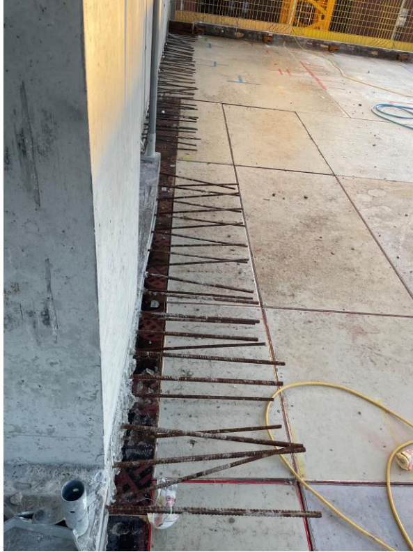
Block D Section C – Reinforcement in place for concrete slab pour
