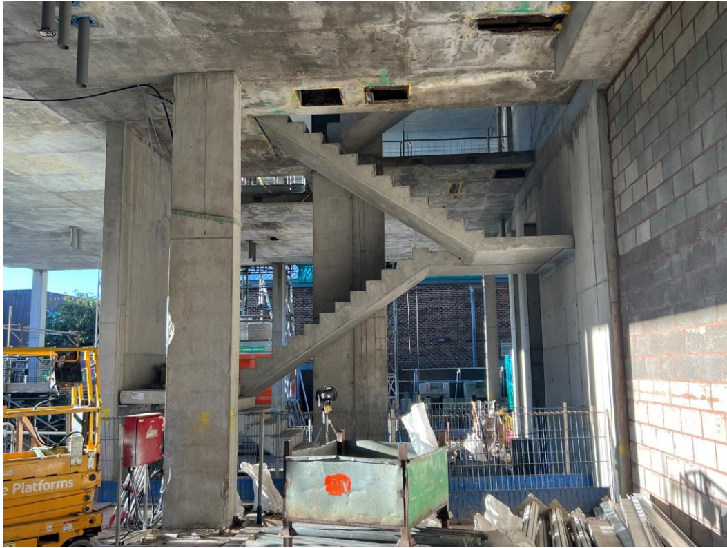
Block D Section B - Pre-cast concrete staircase
