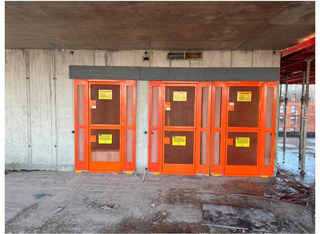
Block D Section A – Temporary lift shaft gates installed
