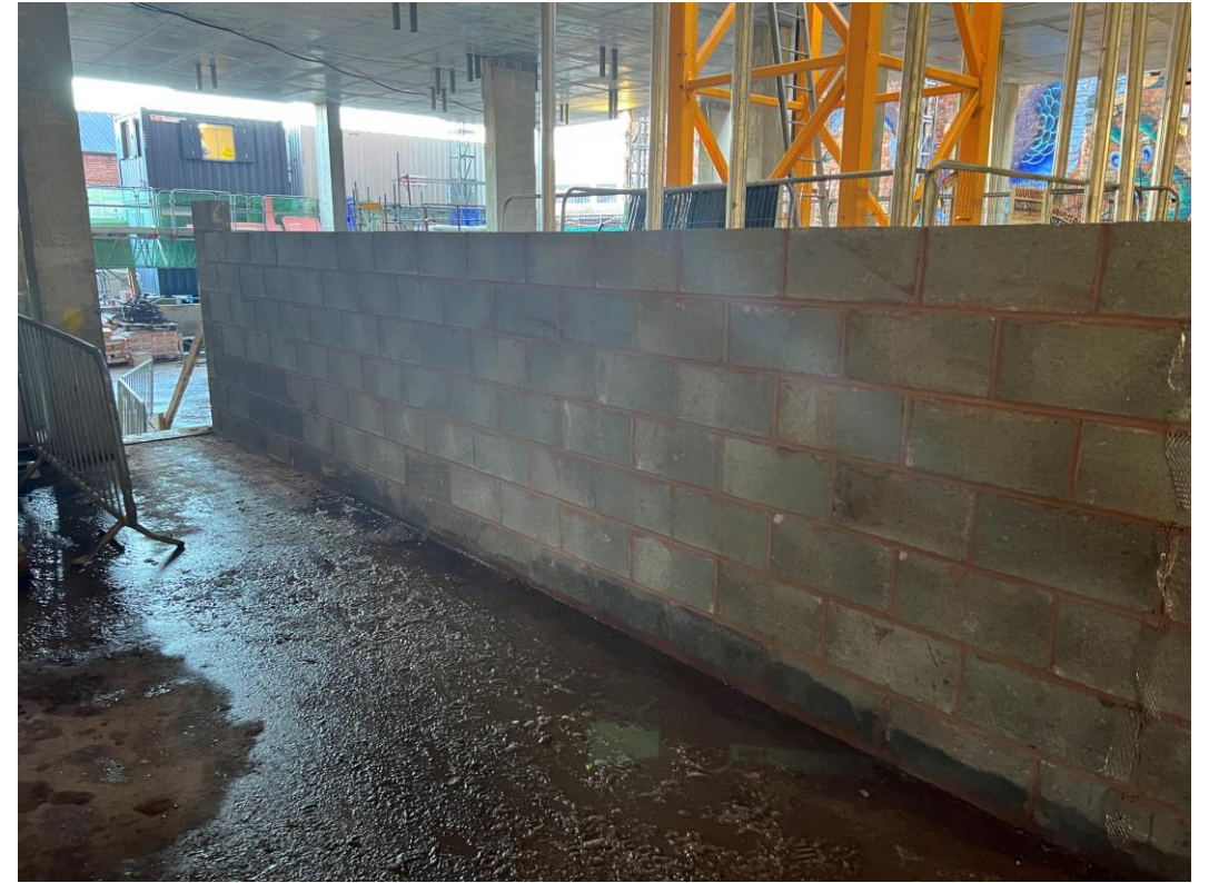
Ground floor masonry walls
