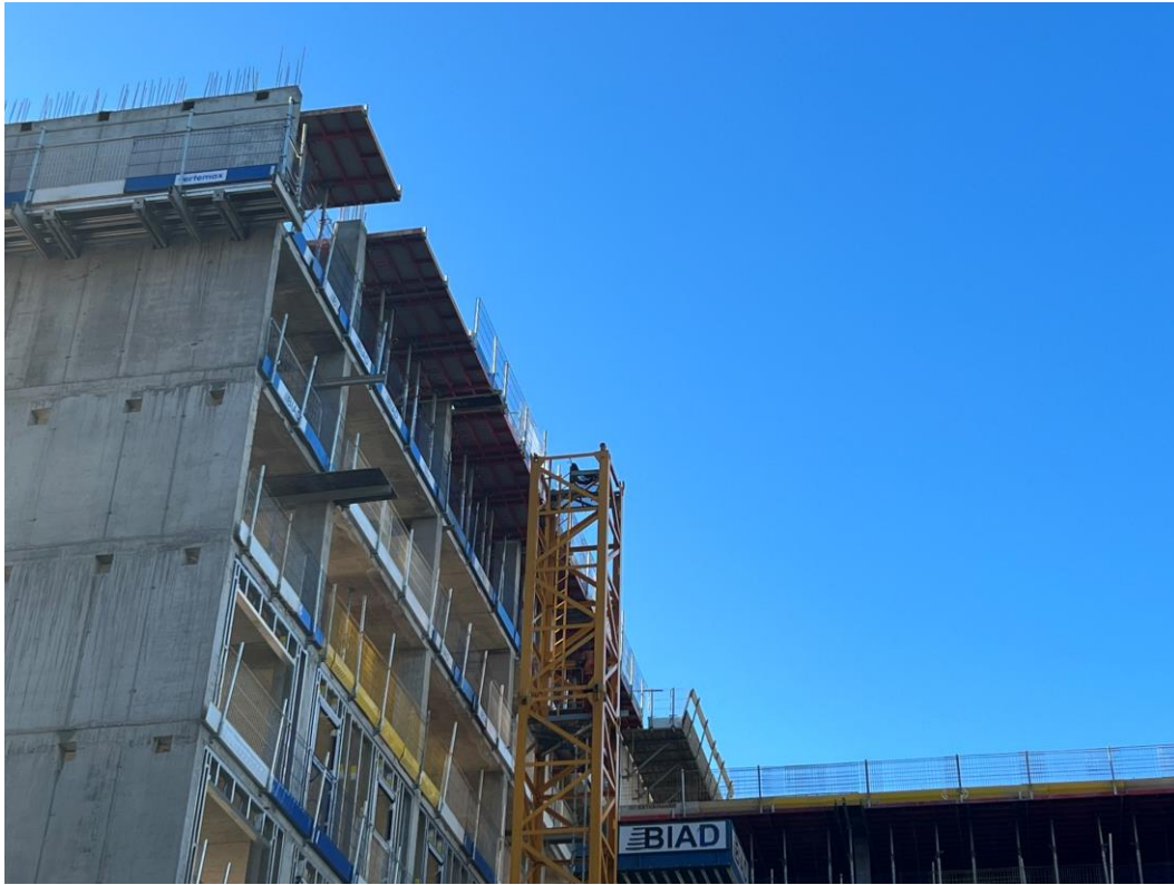
Crane removal ongoing
