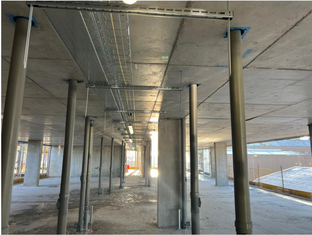
Electrical containment installed has commenced
