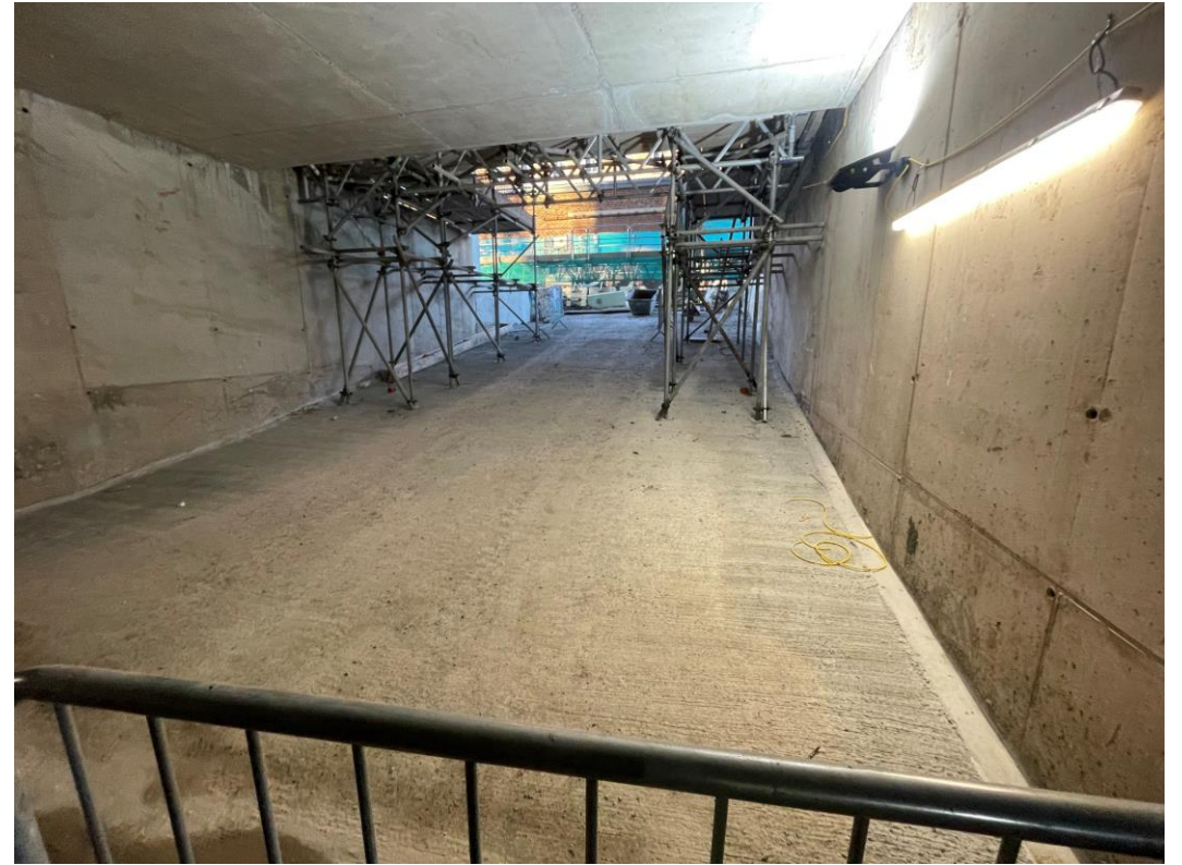
Block D – Basement ramp
