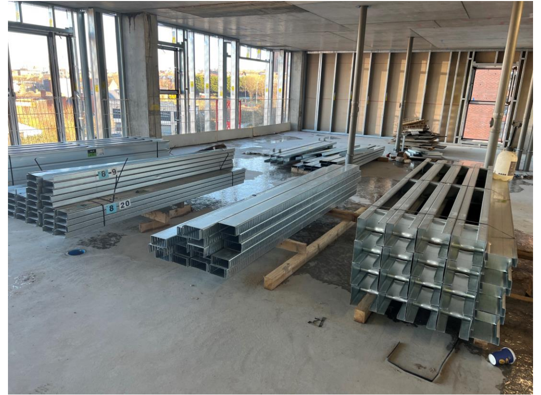
SFS loaded for installation
