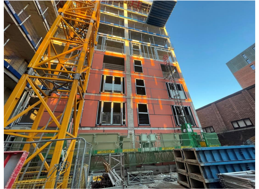
Block D Section A – Weather board installation ongoing
