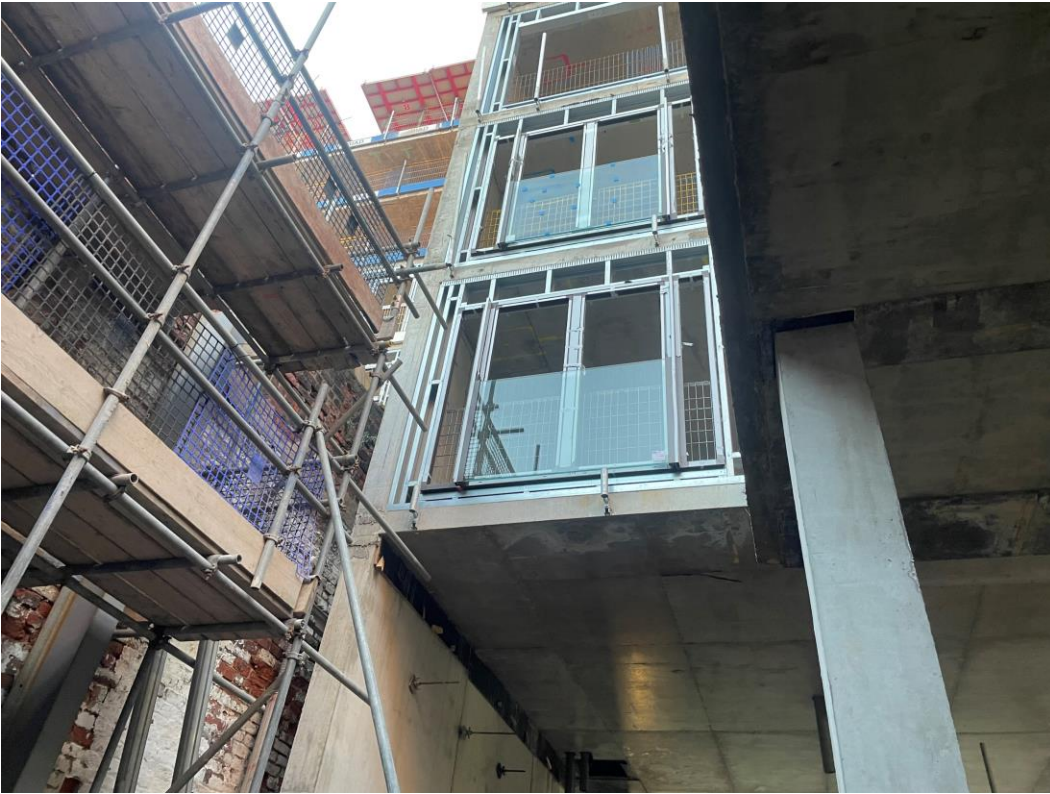
Block D Section B – Glazed balustrade installation commenced
