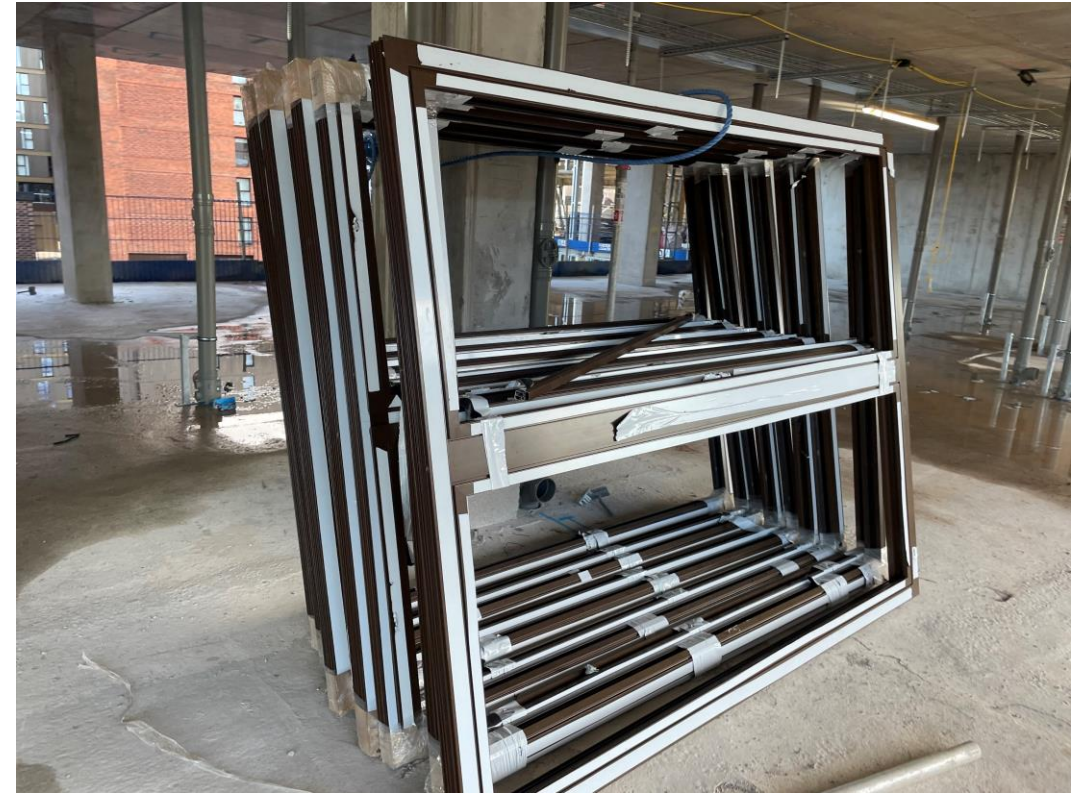
External windows on site
