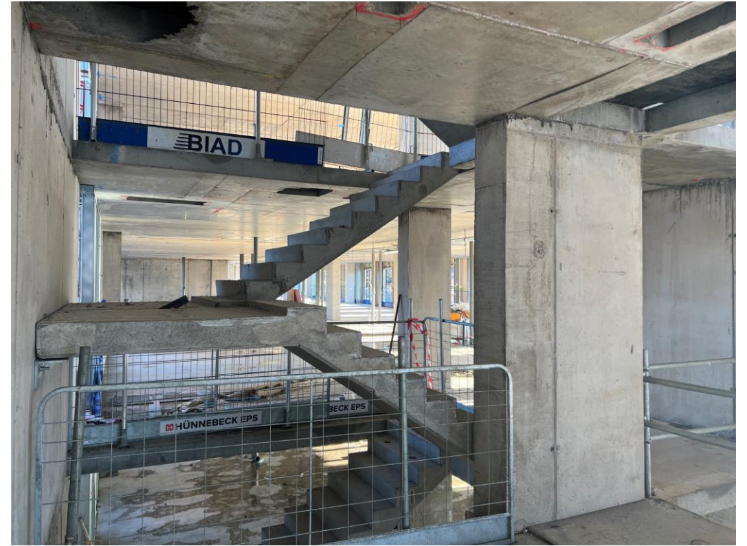
Block D Section B - Pre-cast concrete staircase
