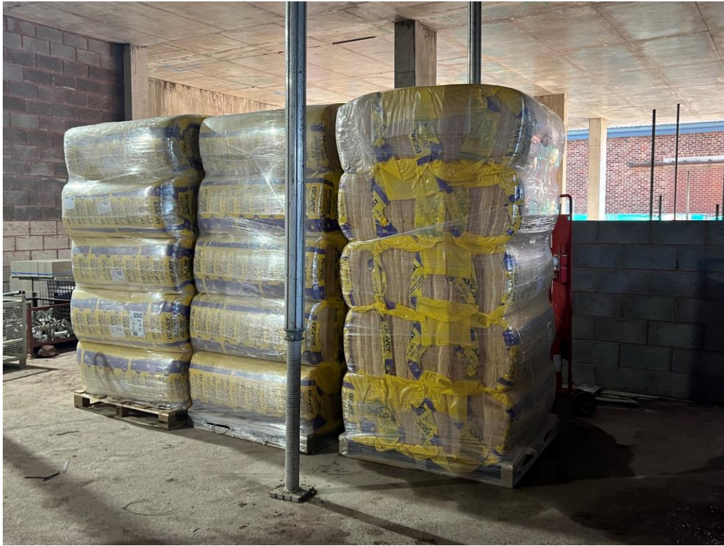
Insulation on site
