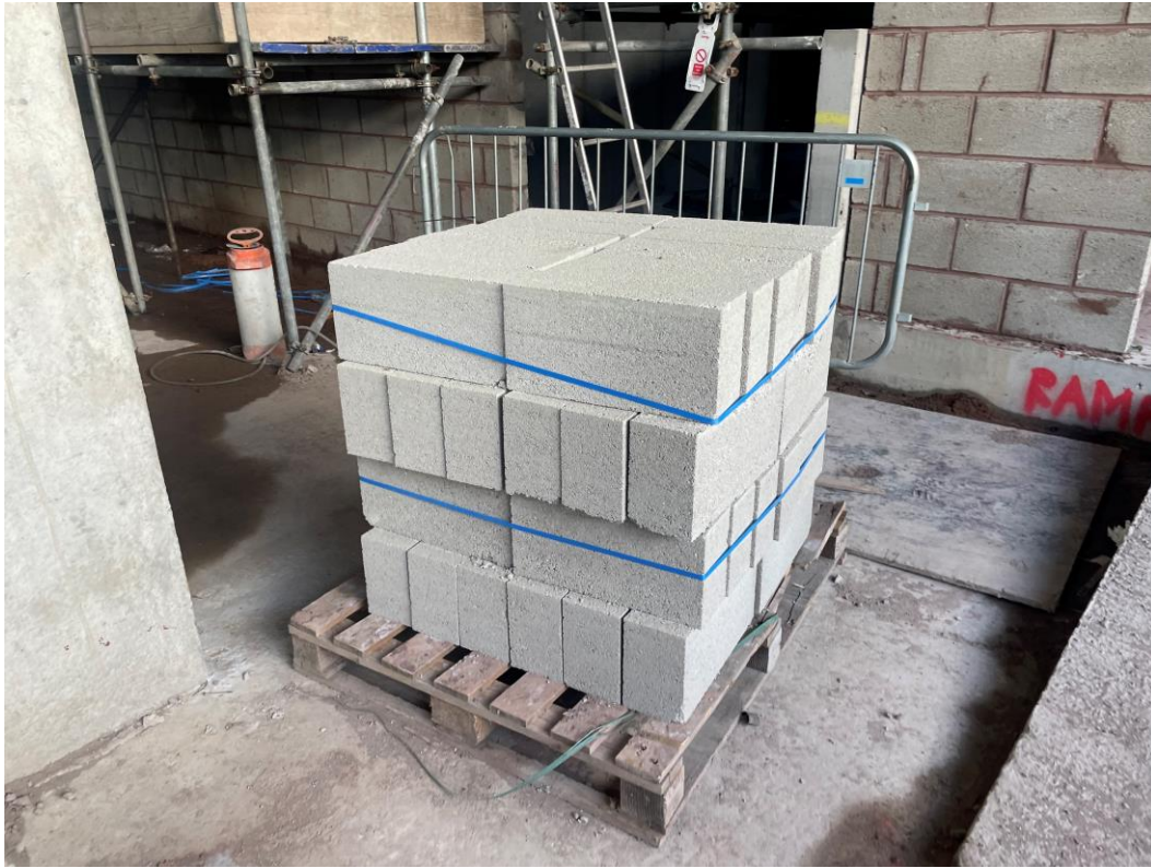
Blockwork loaded for installation
