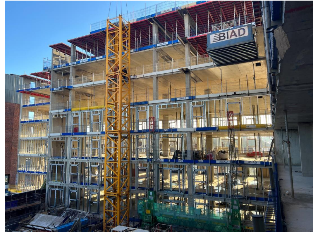
Crane removal ongoing
