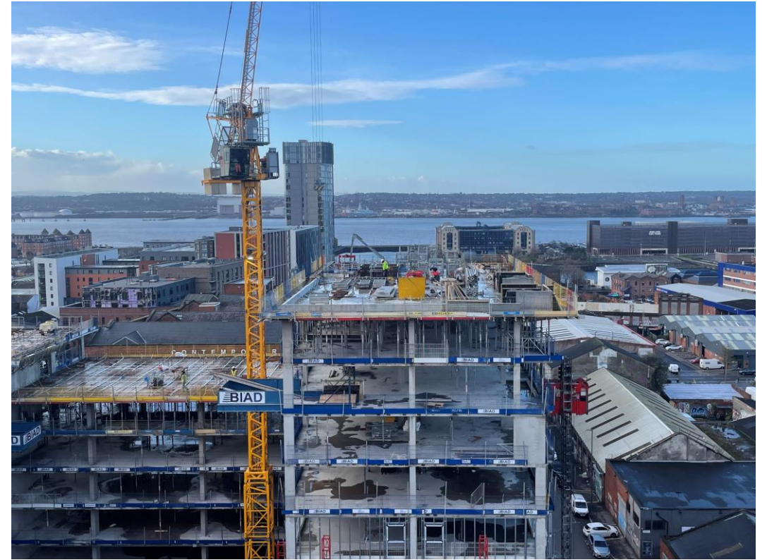
Block D Section A – Viewed from Block B
