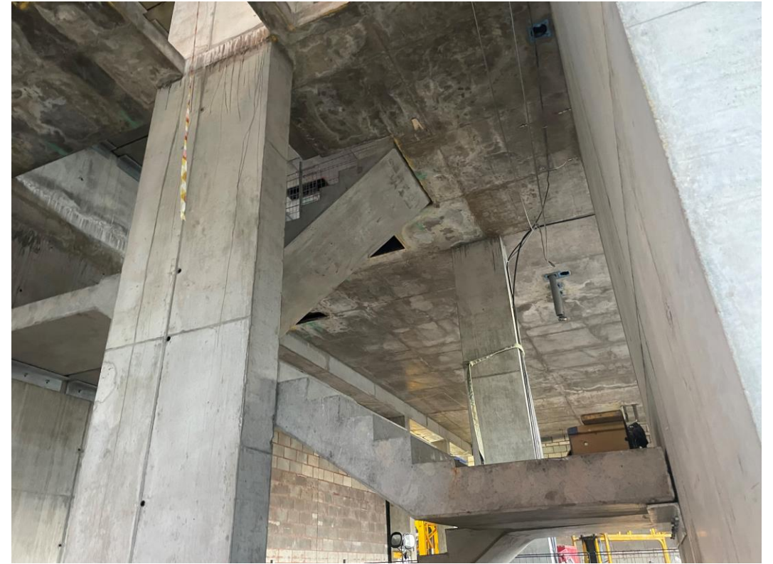
Block D Section B - Pre-cast concrete staircase
