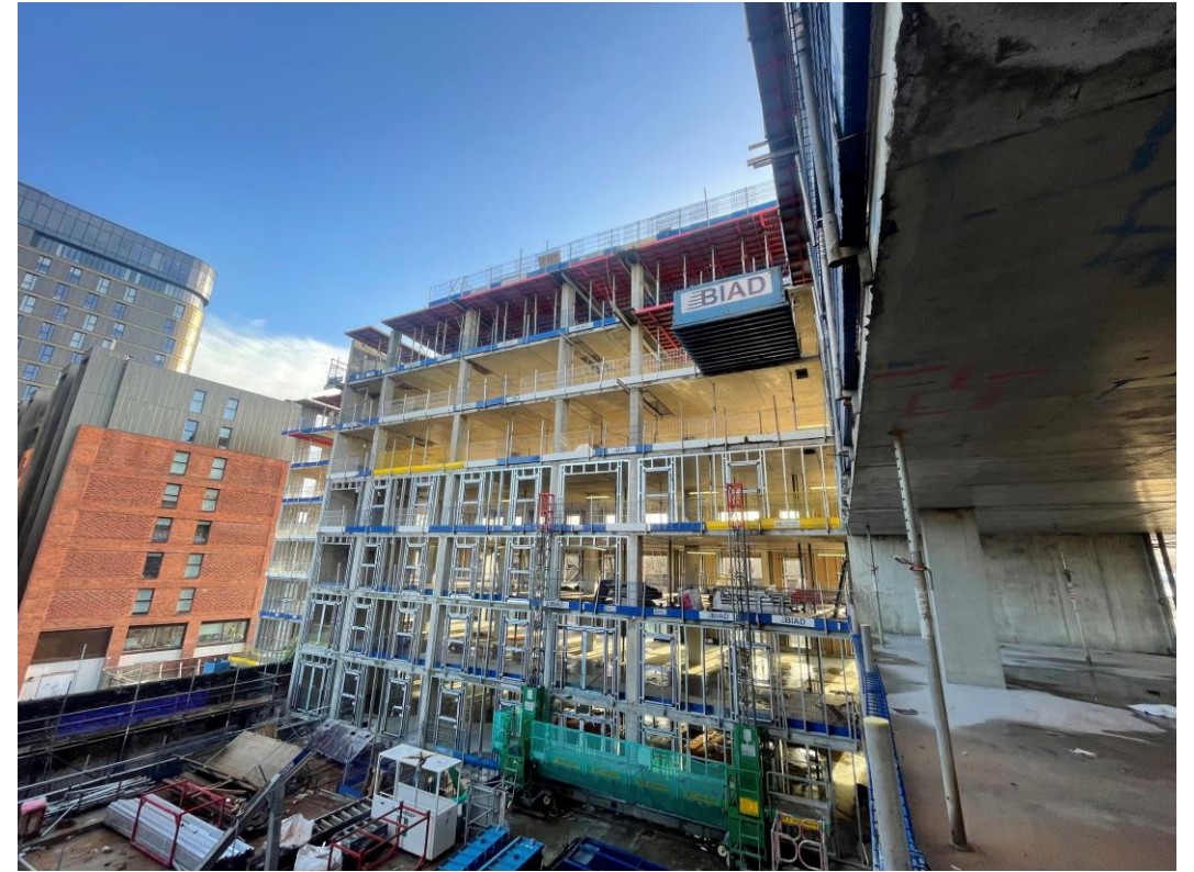
Block D Section B – Viewed from Section C
