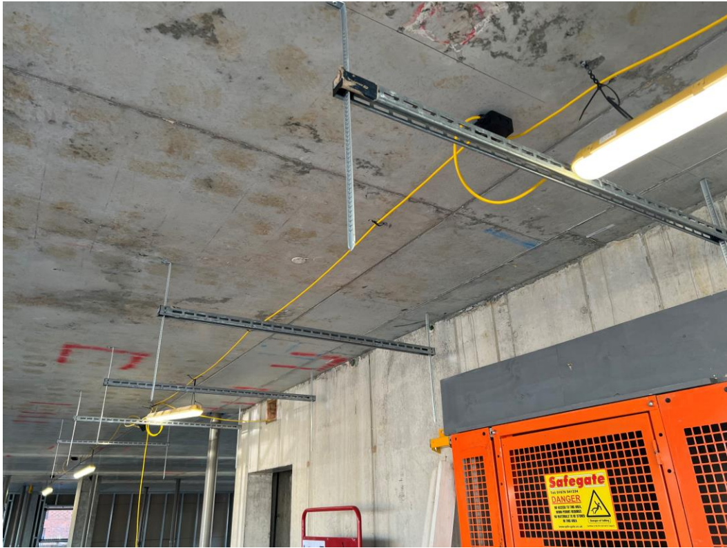
Electrical containment installed has commenced
