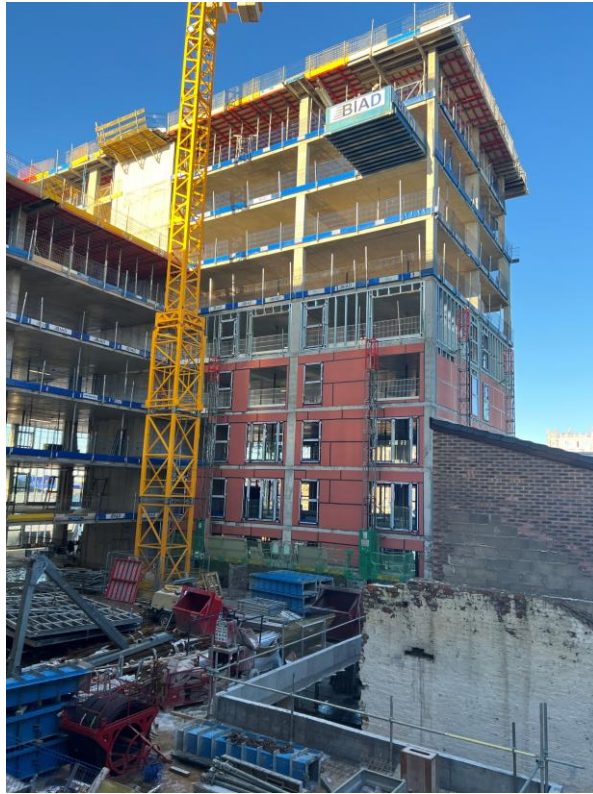
Block D Section A – Weather board installation ongoing
