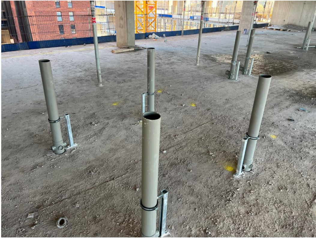
Block D Section C – Soil vent pipes installed
