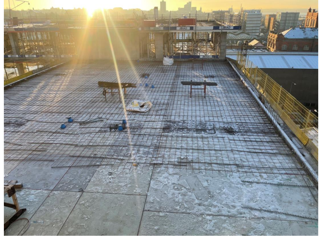
Block D Section C – Reinforcement in place for concrete slab pour
