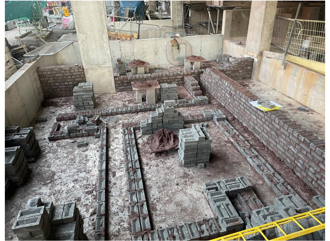
Ground floor masonry walls
