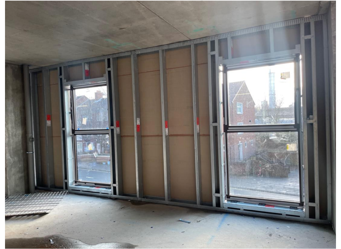
External windows installed
