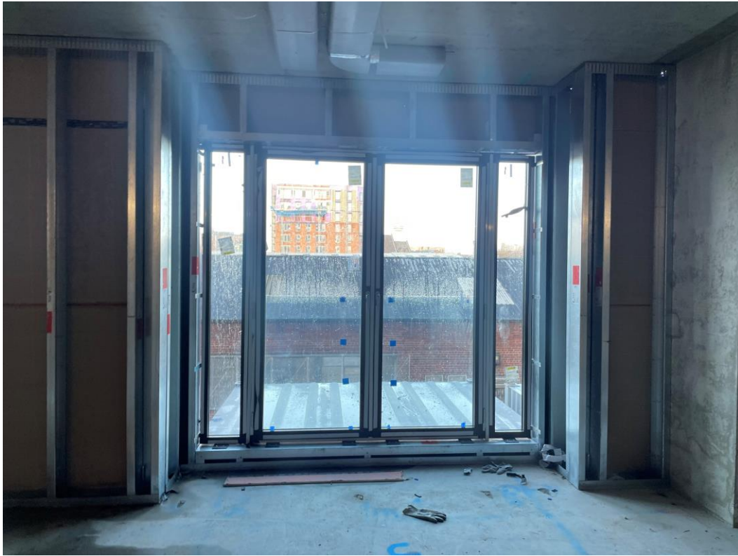
External windows installed
