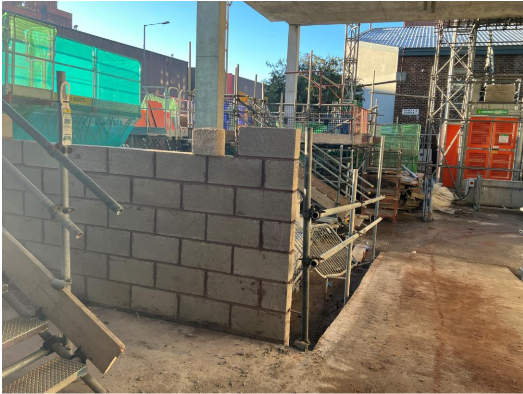
Ground floor masonry walls
