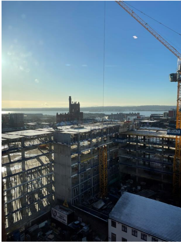
Block D Section B – Viewed from Block B
