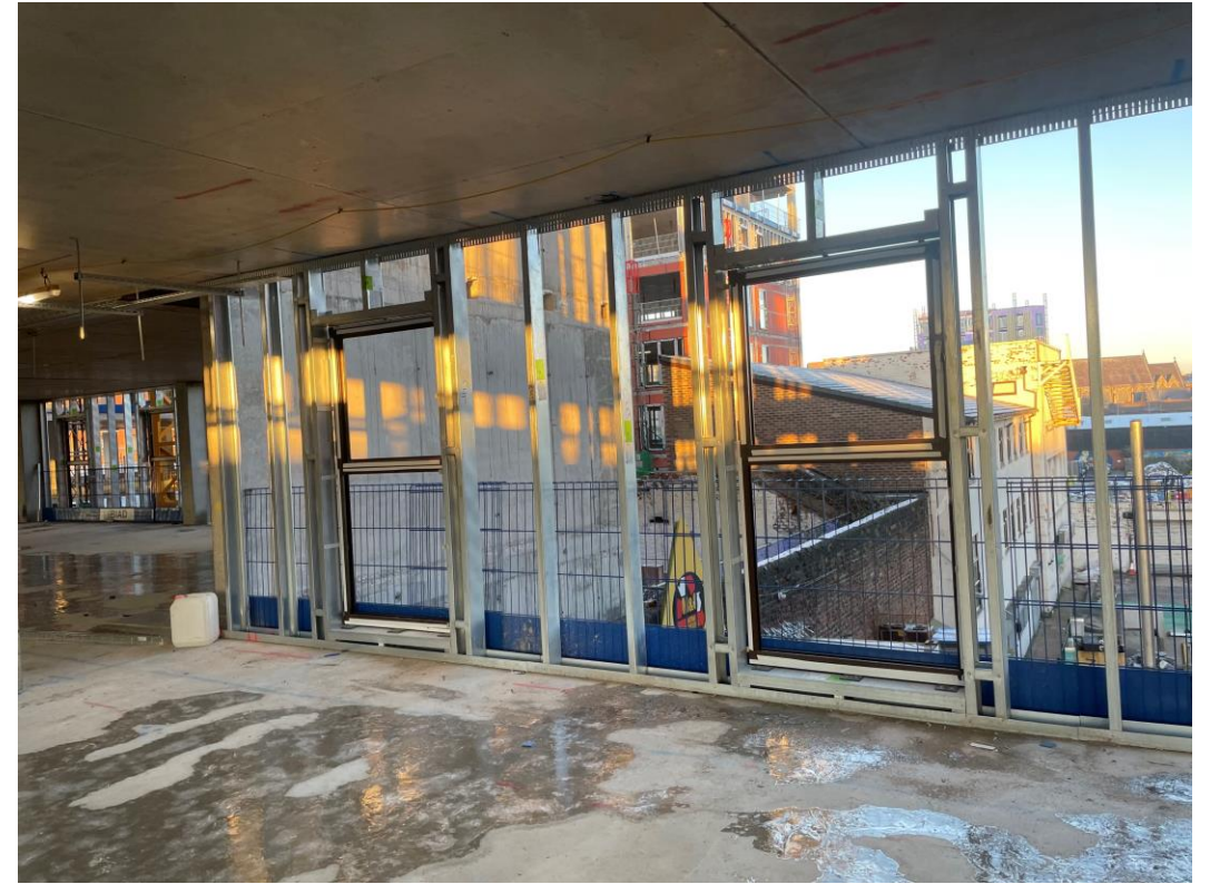
Block D Section B – Window installation ongoing
