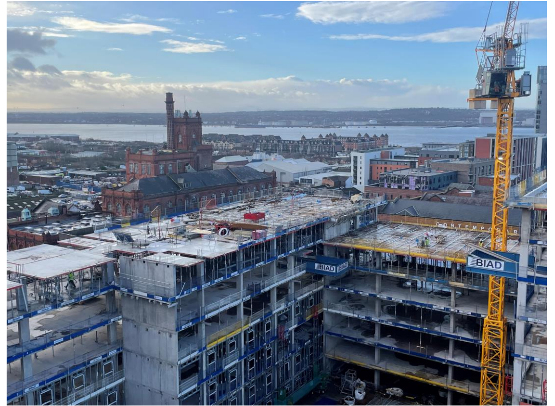
Block D Section B – Viewed from Block B
