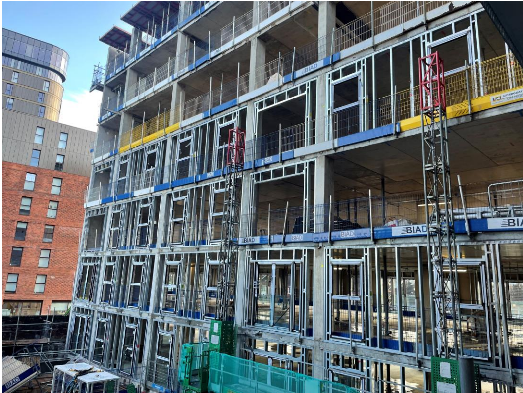
Block D Section B – SFS installation
