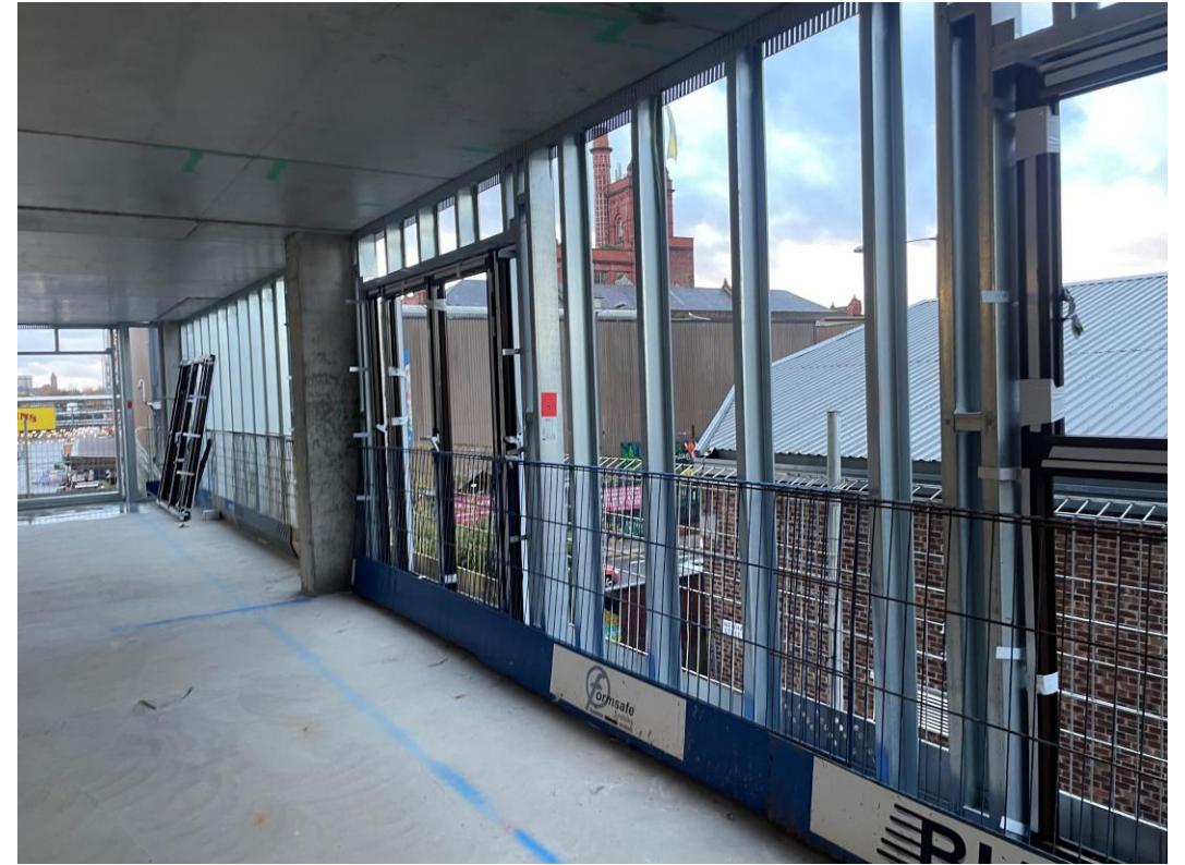
Section B – Window installation commenced
