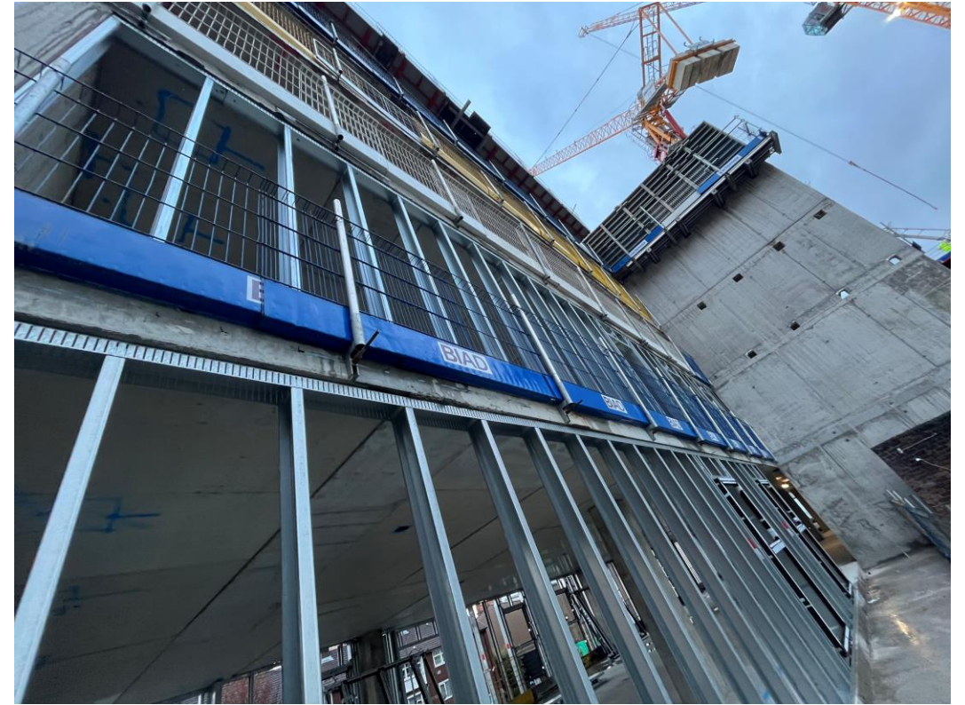
Section A - SFS Installation up to level 4
