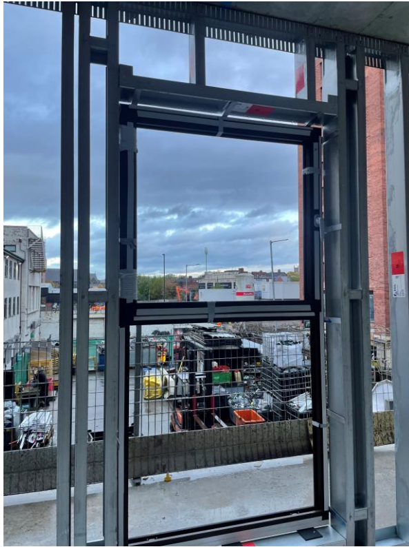
Section B – Window installation commenced
