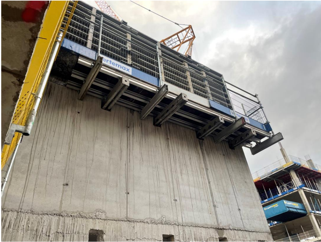
Formwork supports in place
