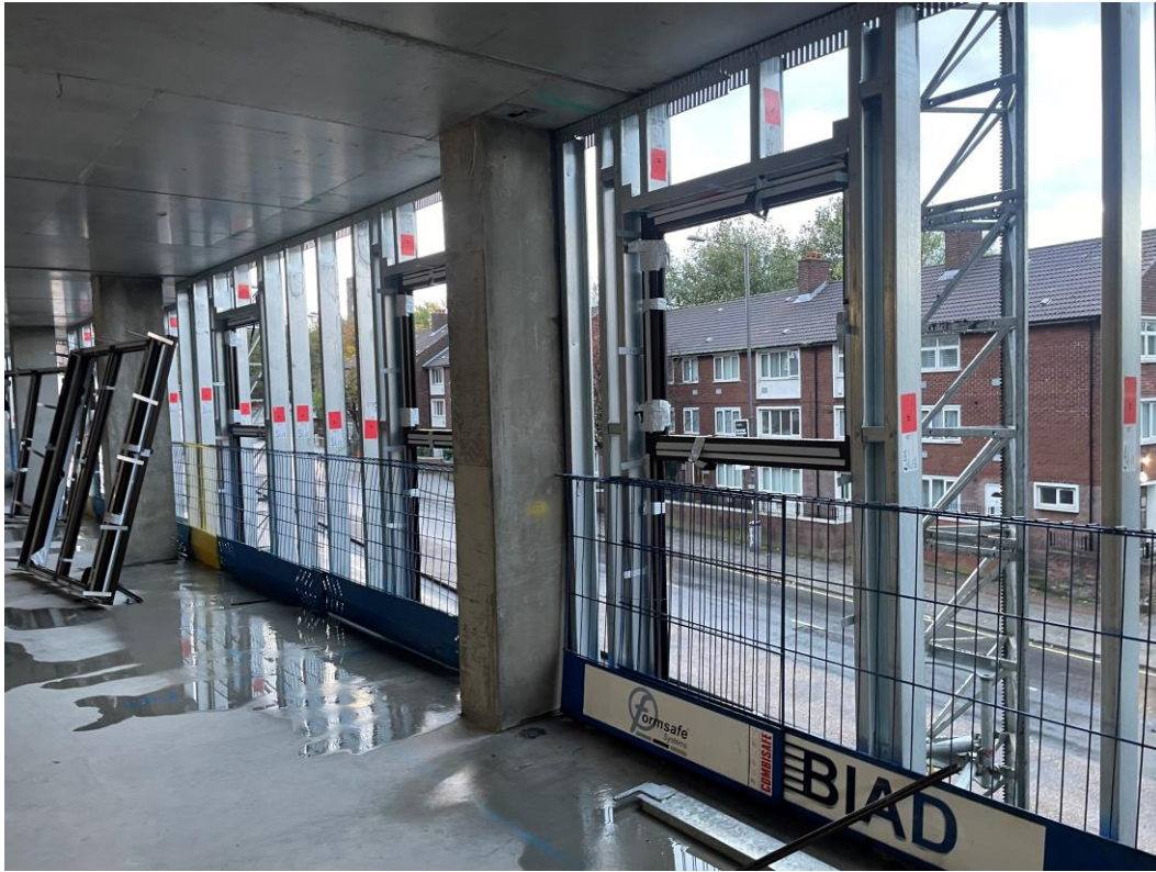
Section B – Window installation commenced
