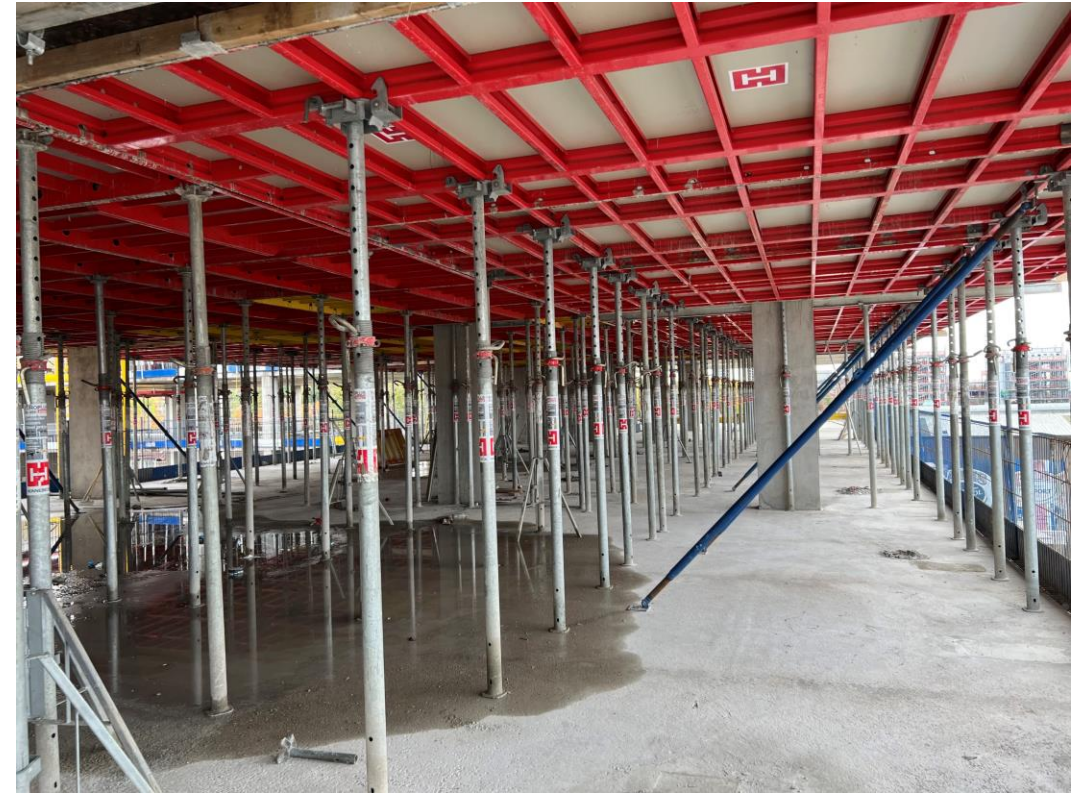
Section C - Table form work in place for Level 5 concrete pour
