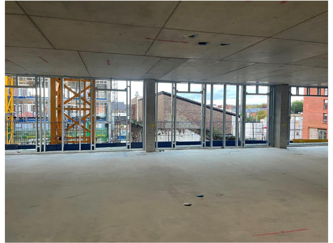
Section B – SFS installation up to level 2
