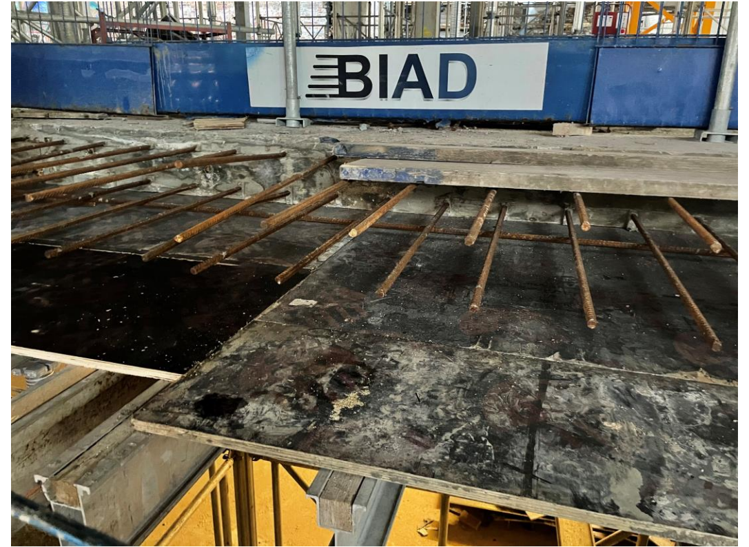
Section A – Concrete slab installation ongoing
