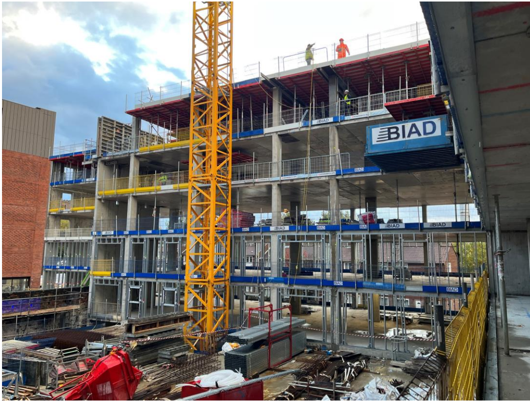
Section B – SFS Installation up to level 2
