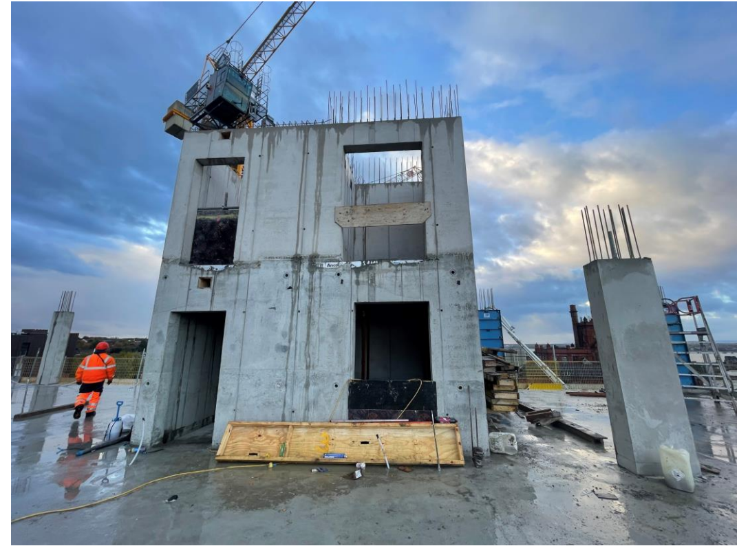
Section A – Concrete frame construction ongoing
