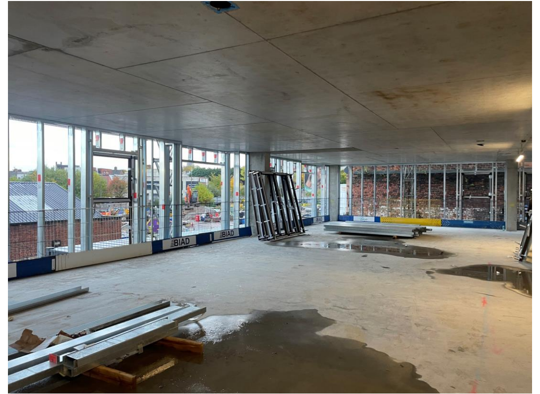
Section A – Window installation commenced
