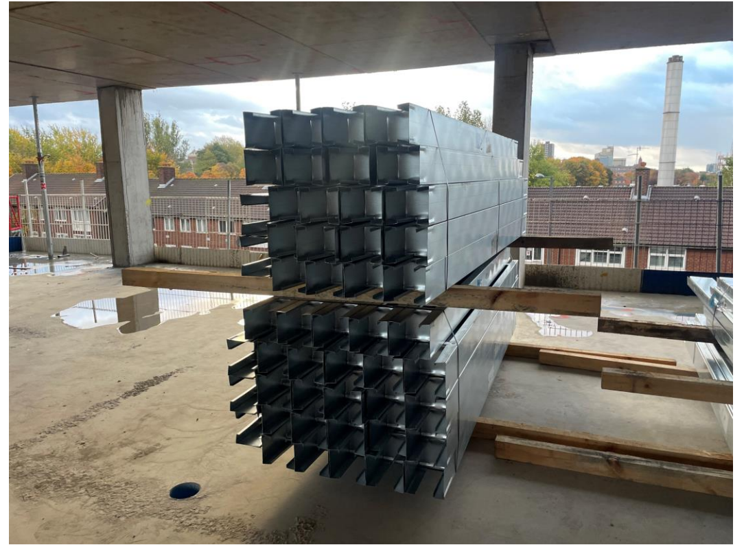
SFS onsite for installation
