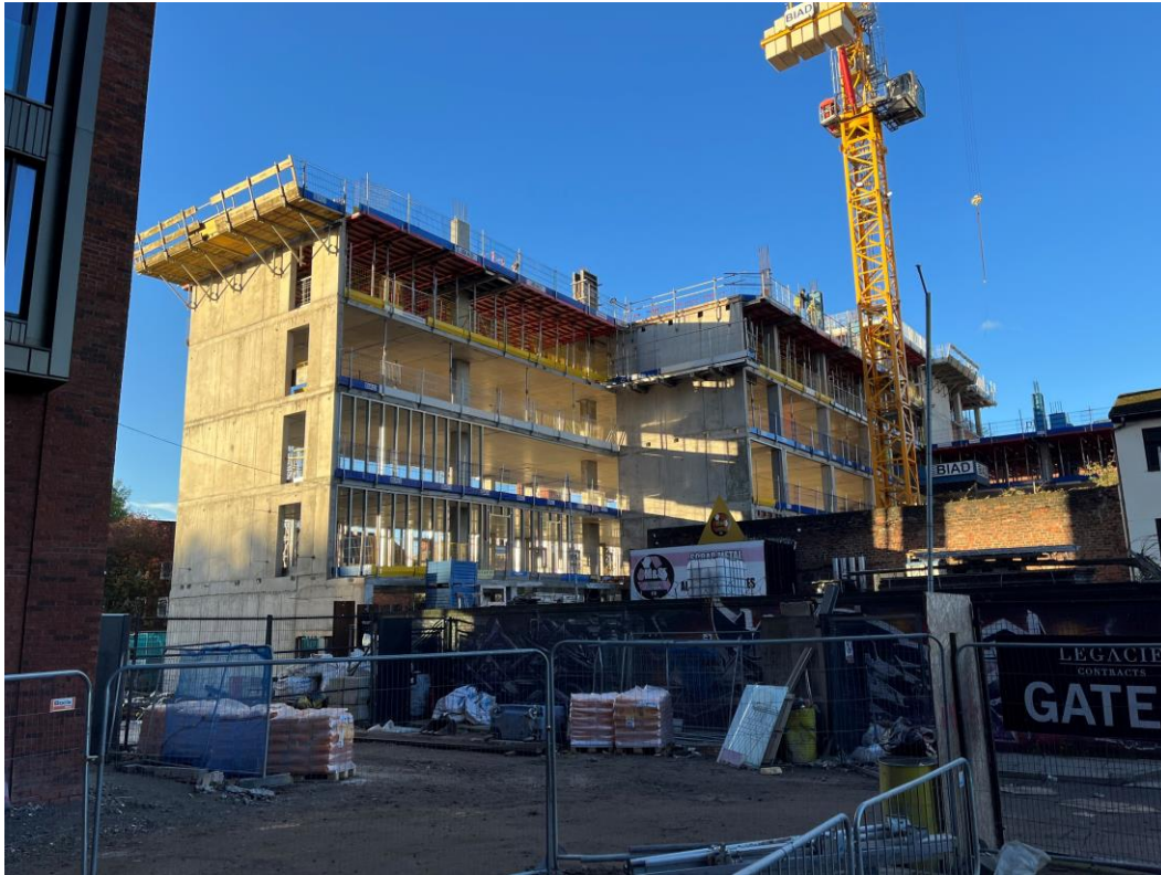
Section B – Viewed from Block B
