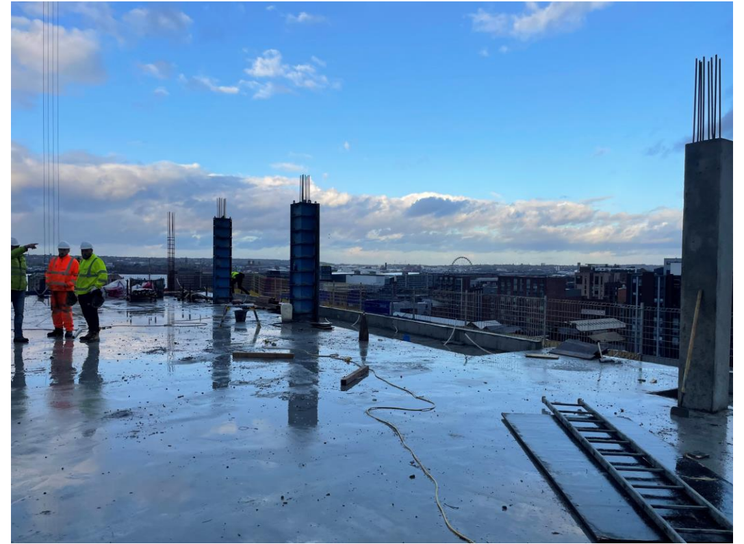
Section A – Concrete frame construction ongoing
