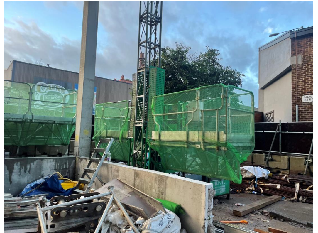
Mast climbers installed
