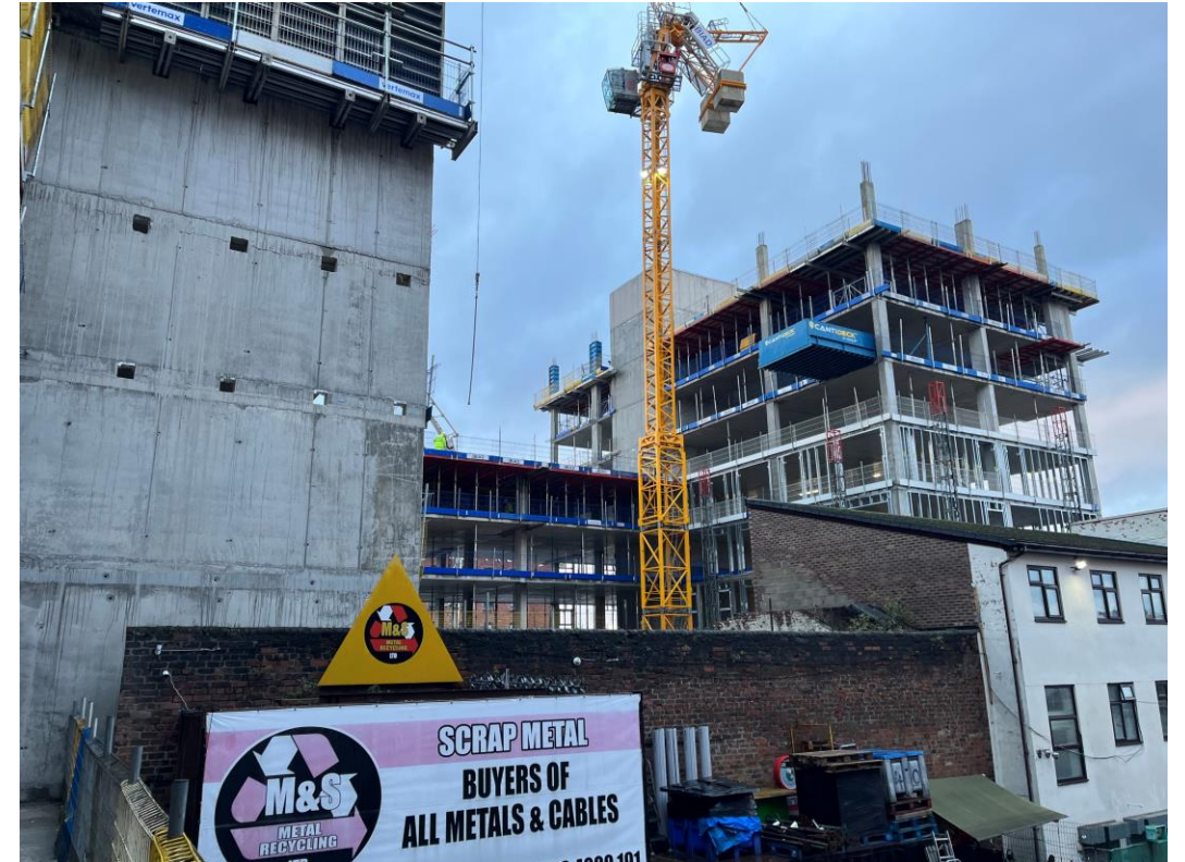
Concrete frame construction ongoing
