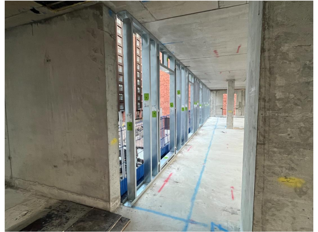
Section B - SFS Installation up to level 2
