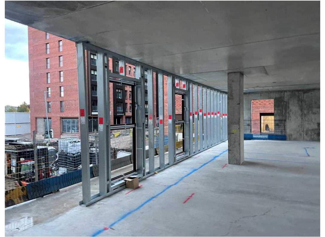
Section B – Window installation commenced
