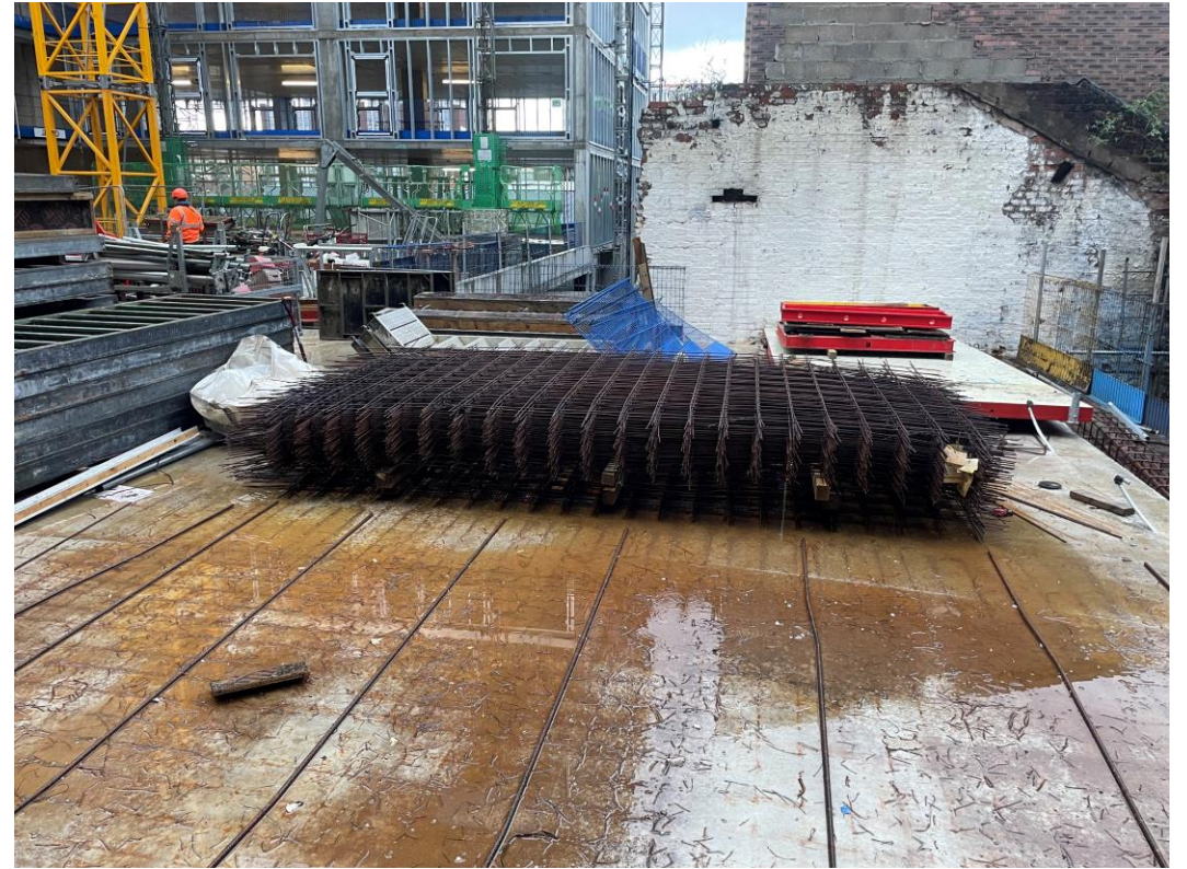
Reinforcement onsite for installation
