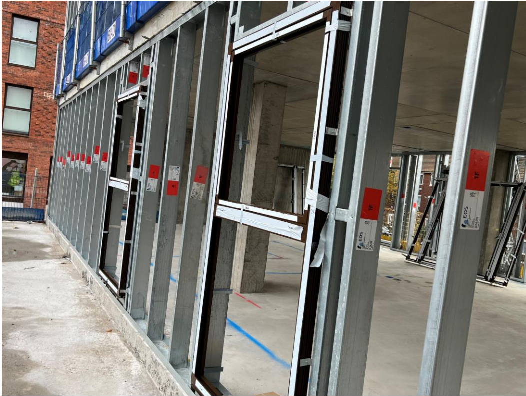
Section B – Window installation ongoing
