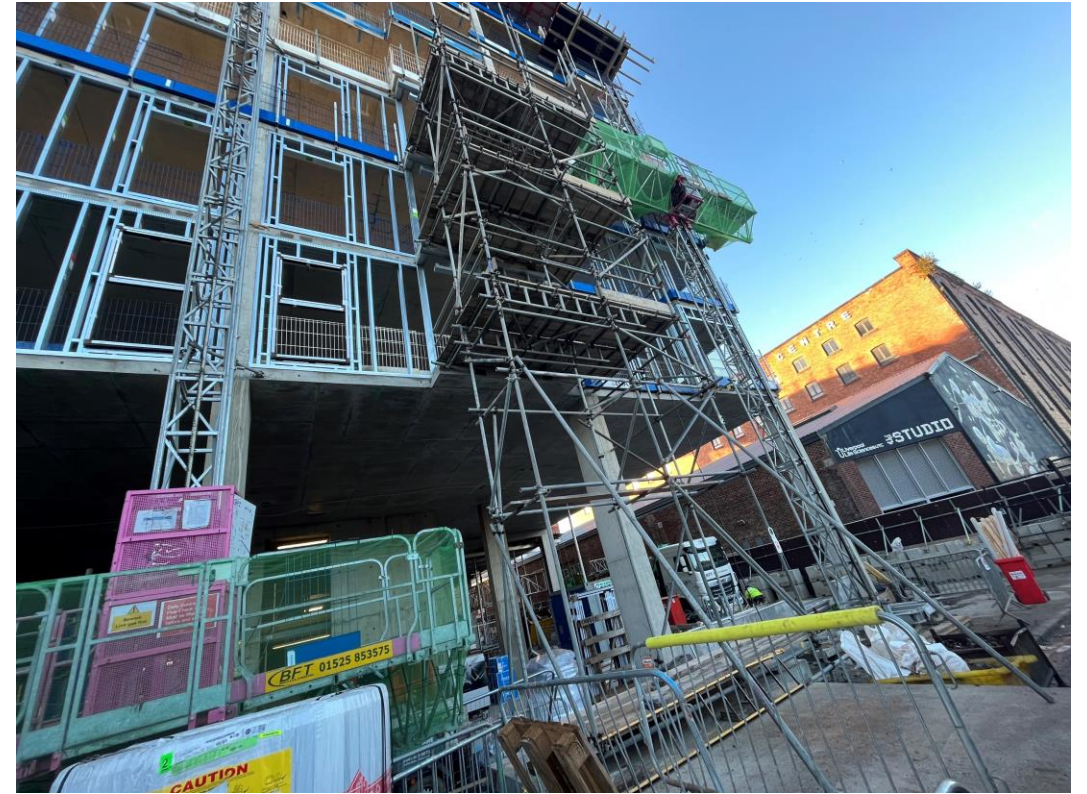
Scaffolding installation ongoing
