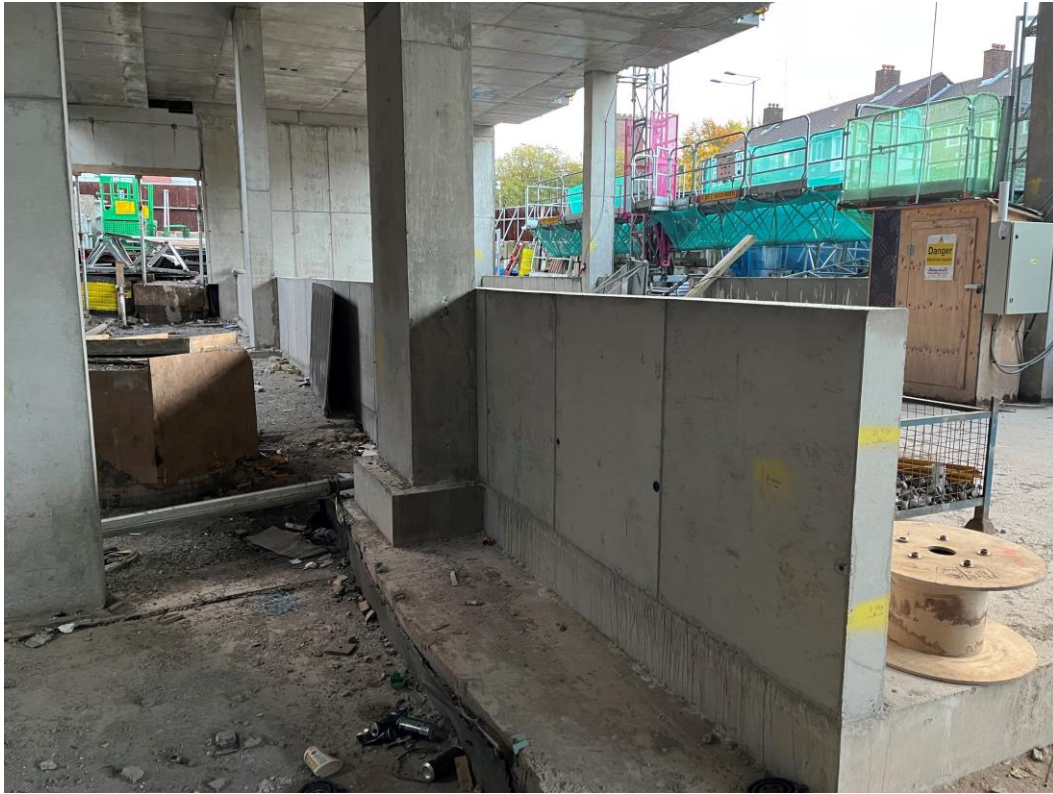
Section B – Concrete upstand formation ongoing
