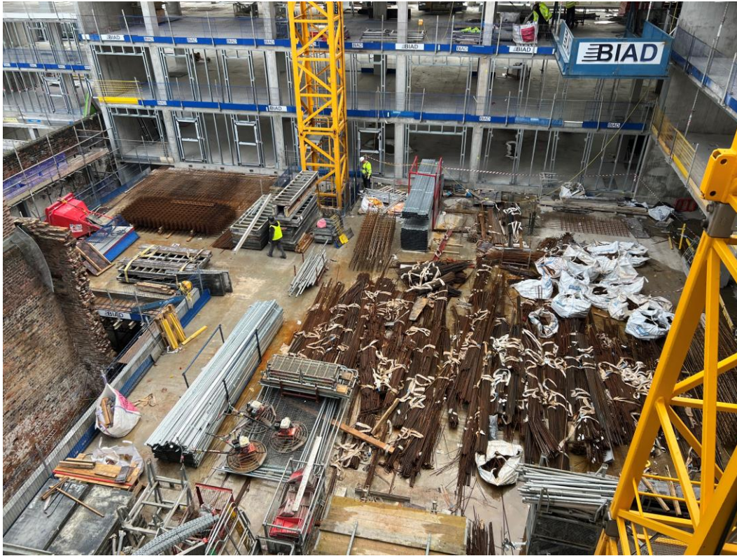
Steel reinforcement onsite for installation
