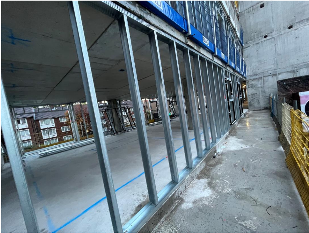
Section B – SFS Installation up to level 2
