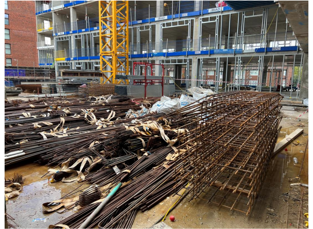
Reinforcement onsite for installation
