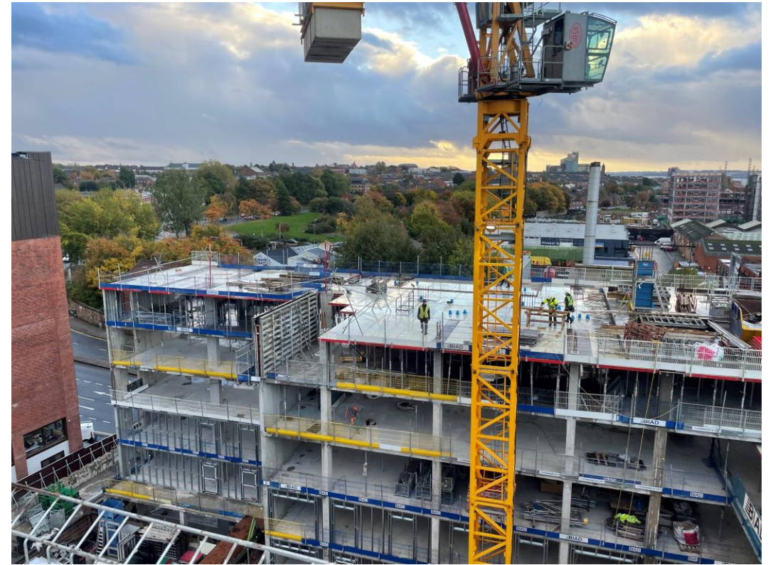
Section B – Preparation works ongoing for Level 6 concrete pour
