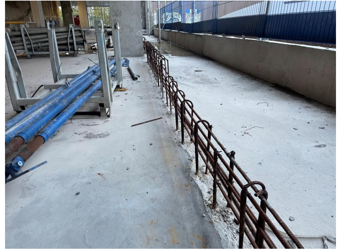
Section C – Reinforcement installed for concrete upstand
