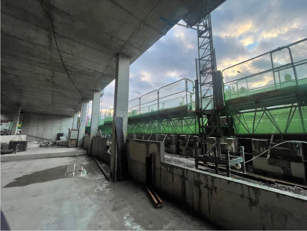
Mast climbers installed
