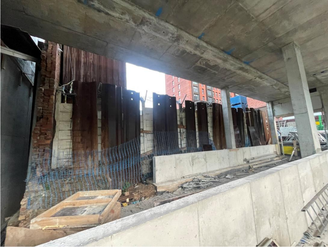
Sheet piles installed
