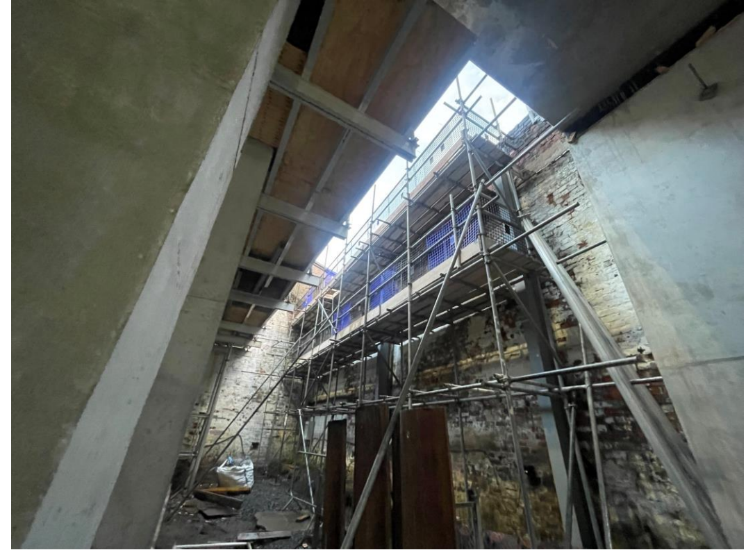
Party wall works
