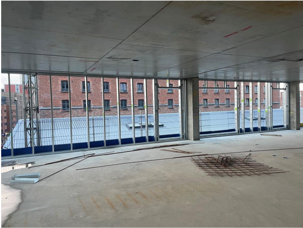
Section B – SFS installation up to level 2
