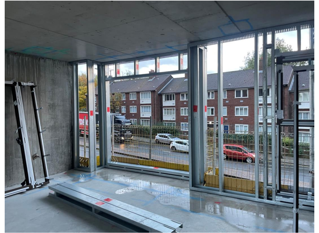
Section B – SFS installation up to level 2
