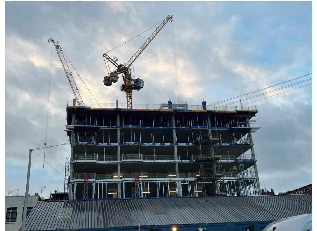
Section A - Concrete frame construction ongoing
