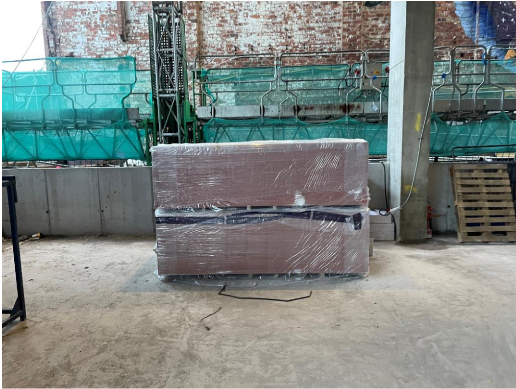
Weatherboard onsite for installation
