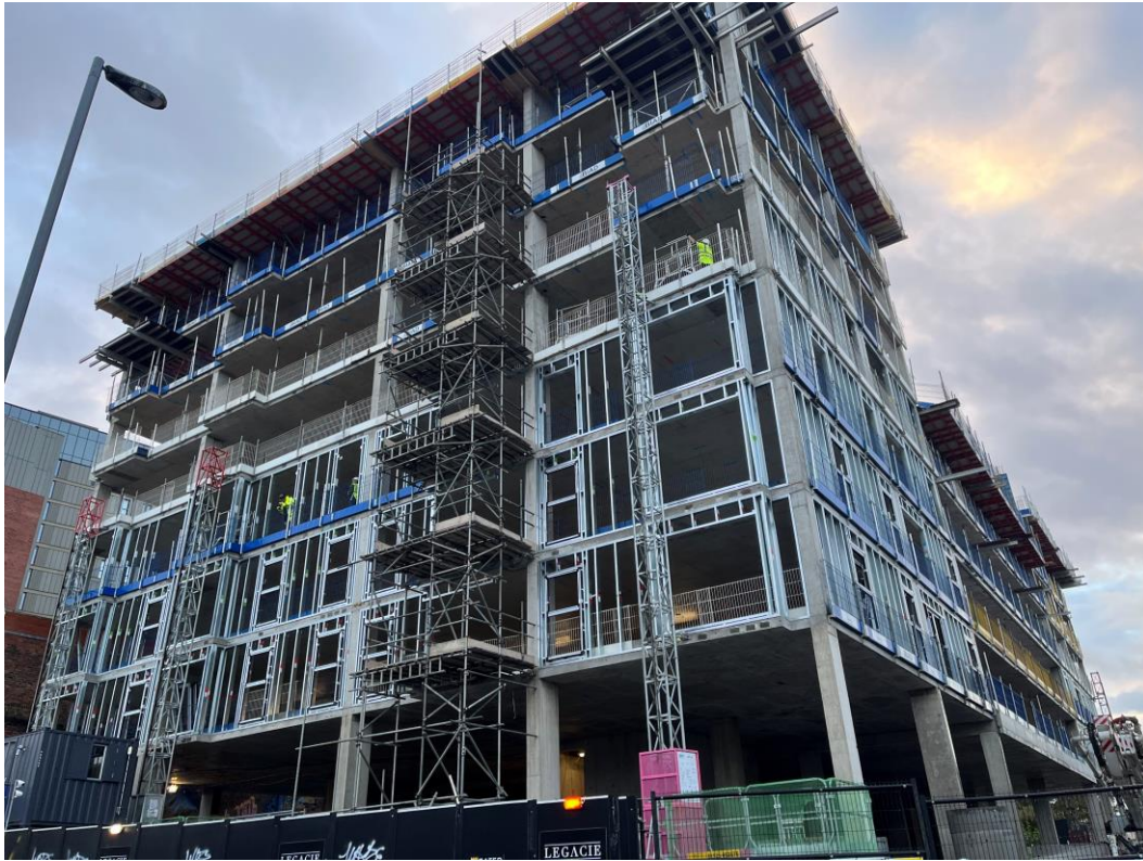
Section A – SFS Installation up to level 4
