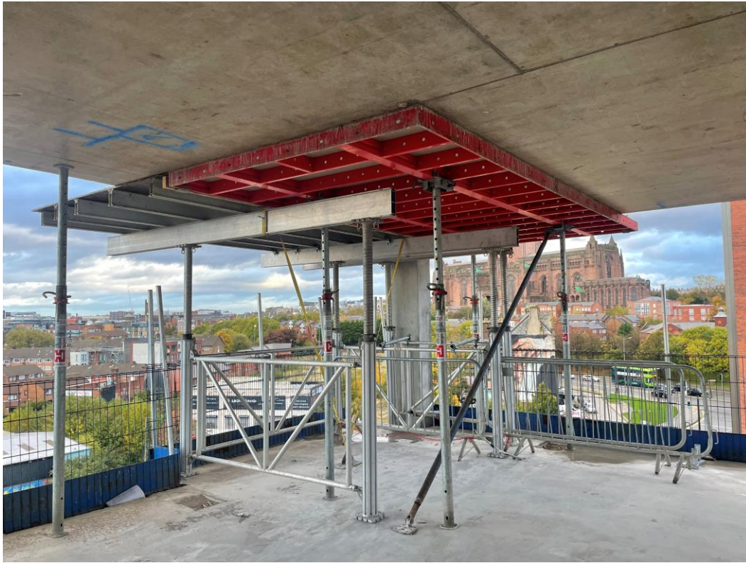
Section A – Removal of form work following level 7 concrete pour
