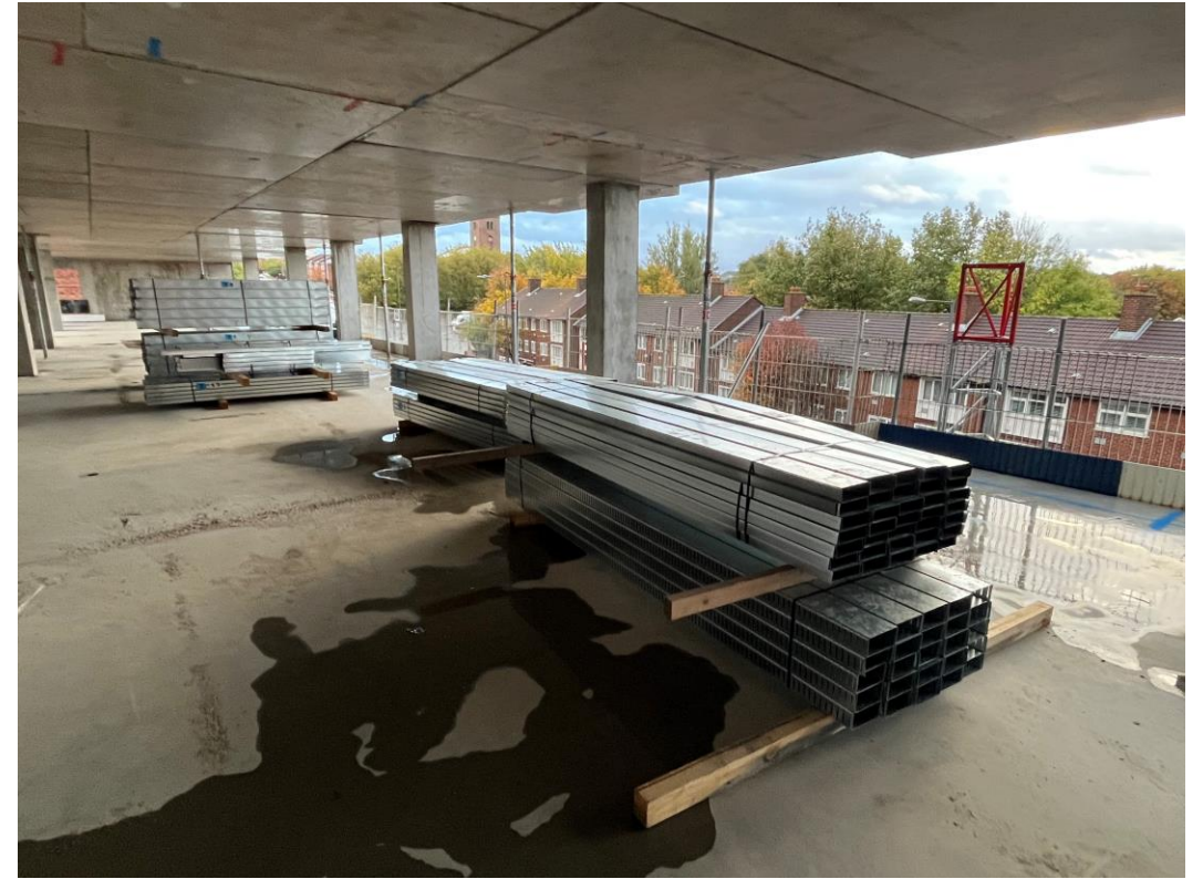
SFS onsite for installation
