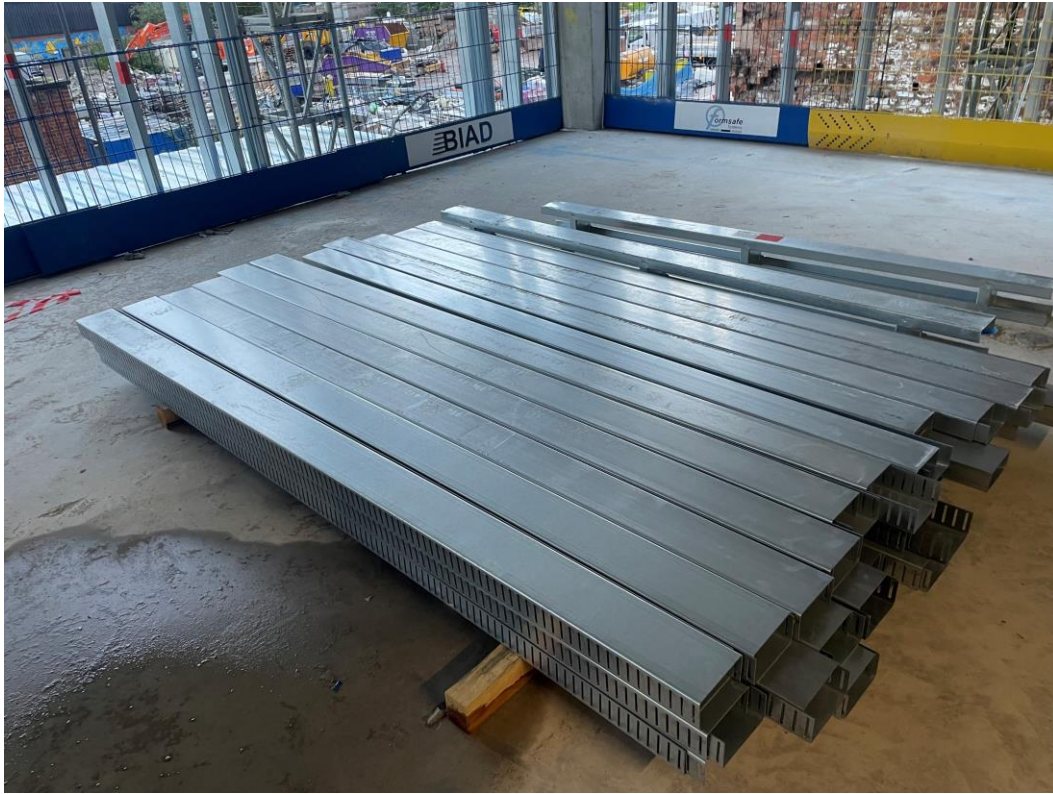
SFS onsite for installation
