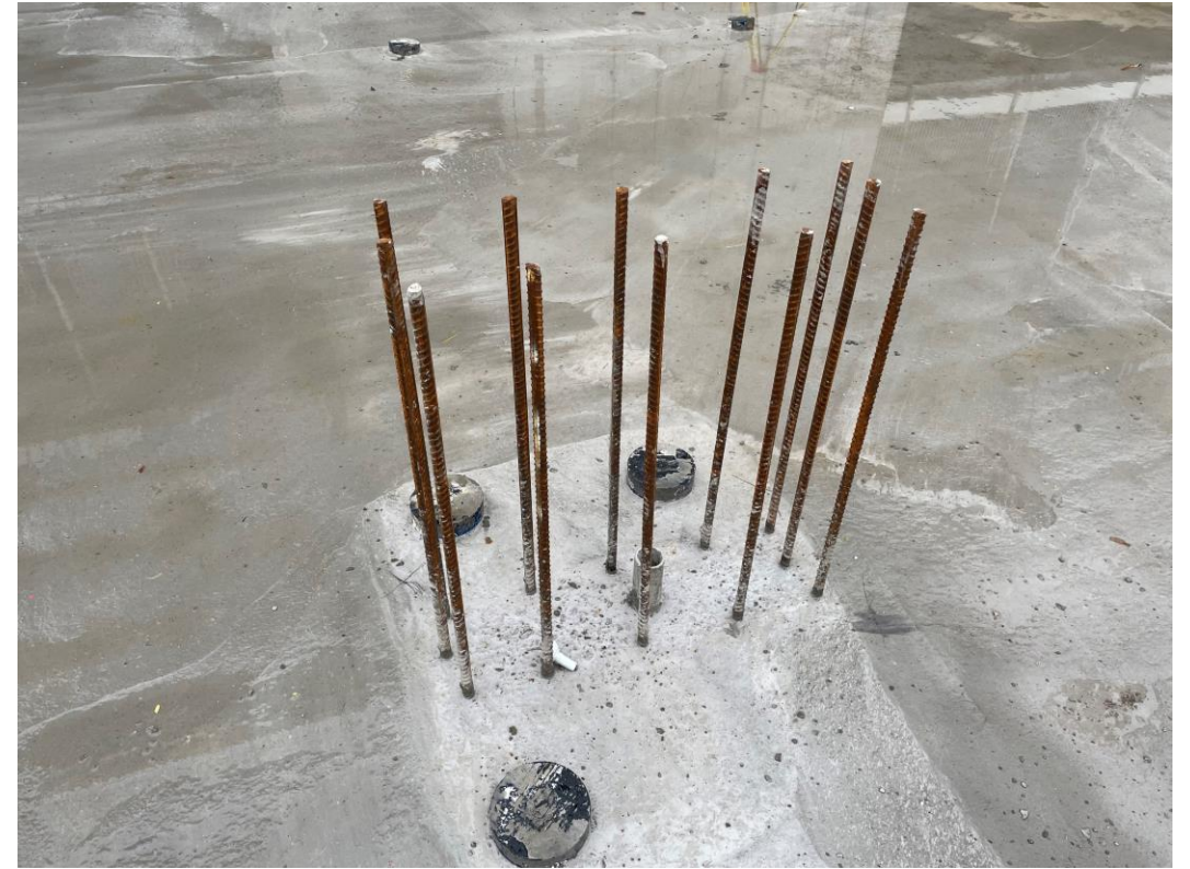
Section C – Column reinforcement
