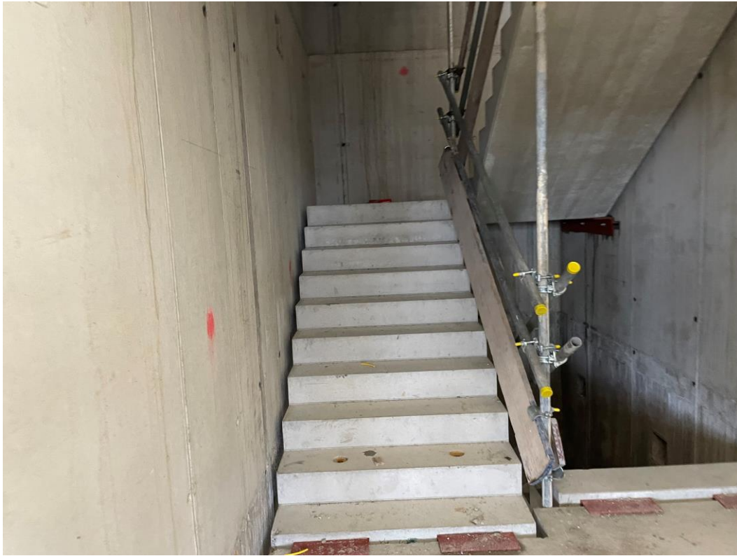
Section A – Concrete stair case installation ongoing
