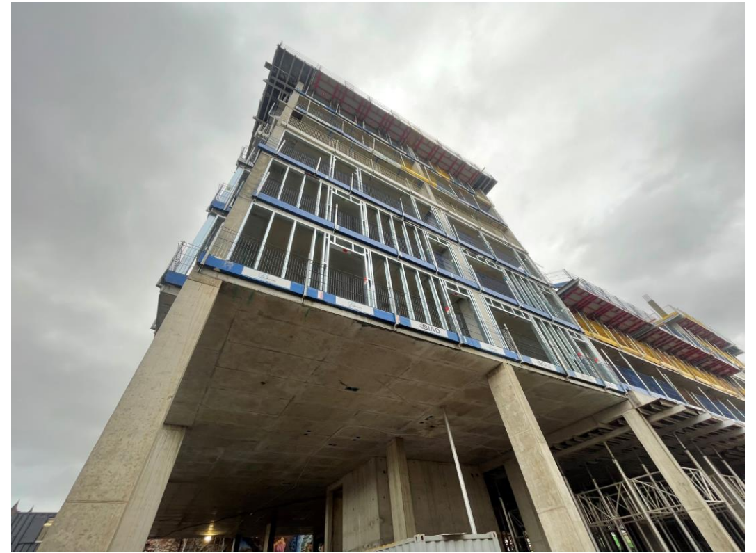
Section A – SFS installation
