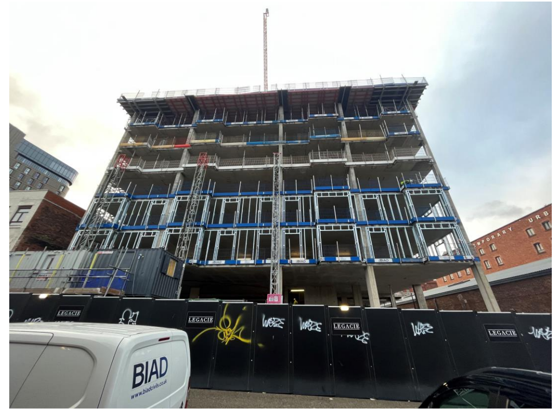
Section A – SFS installation commenced
