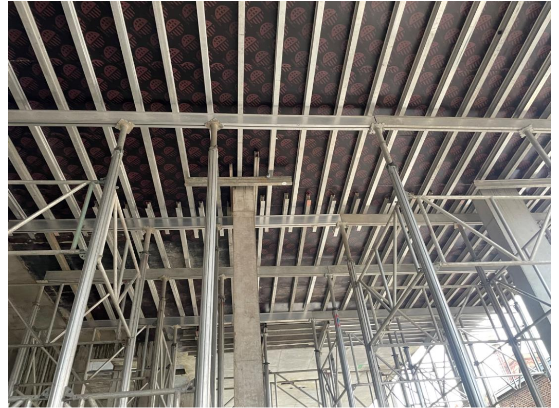
Section C – Formwork in place
