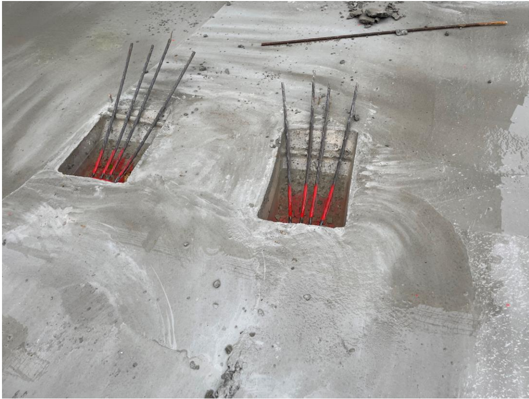
Section C – Installation of PT Strands
