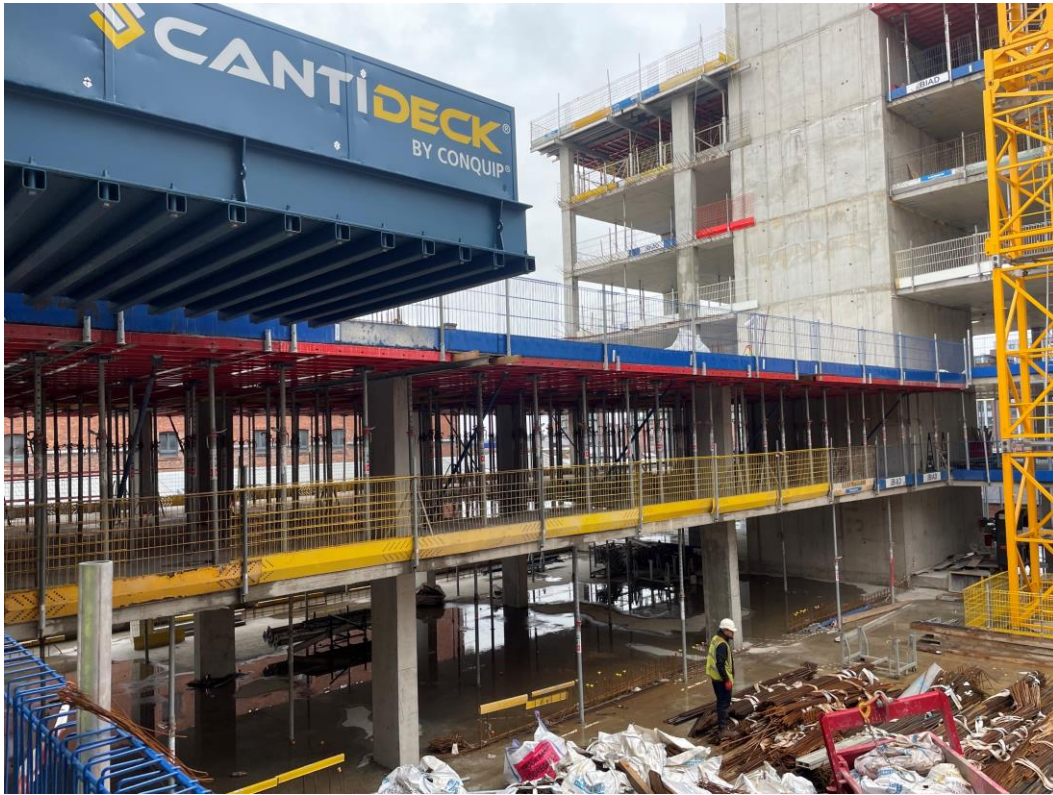
Section C – Formwork in place following Level 3 pour
