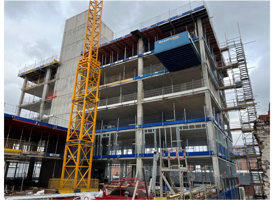
Section A – Concrete frame construction ongoing
