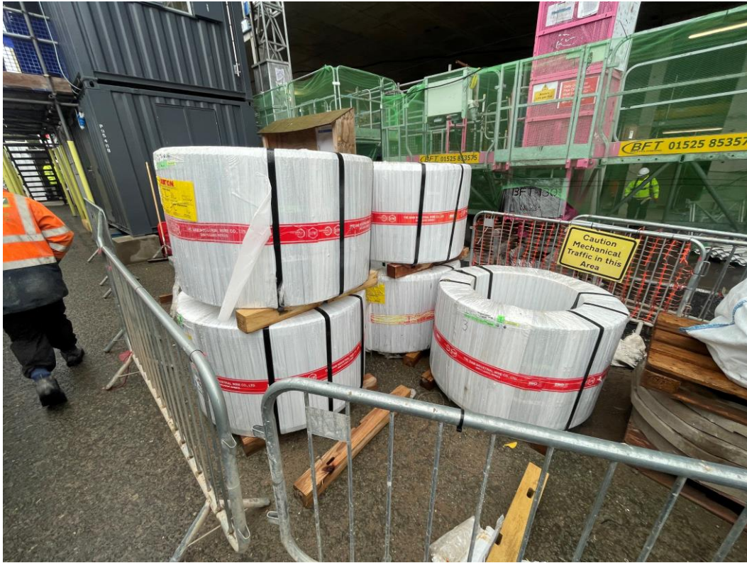
PT Strand onsite for installation
