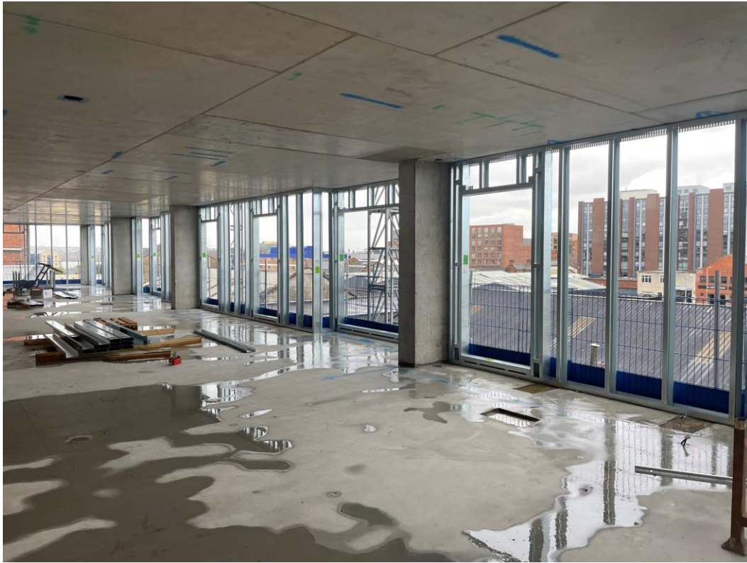
Section A – SFS Installation commenced
