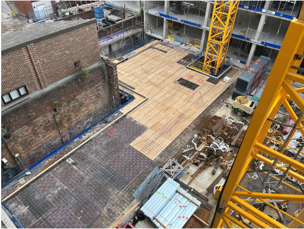
Section C – Preparations made for Podium concrete pour
