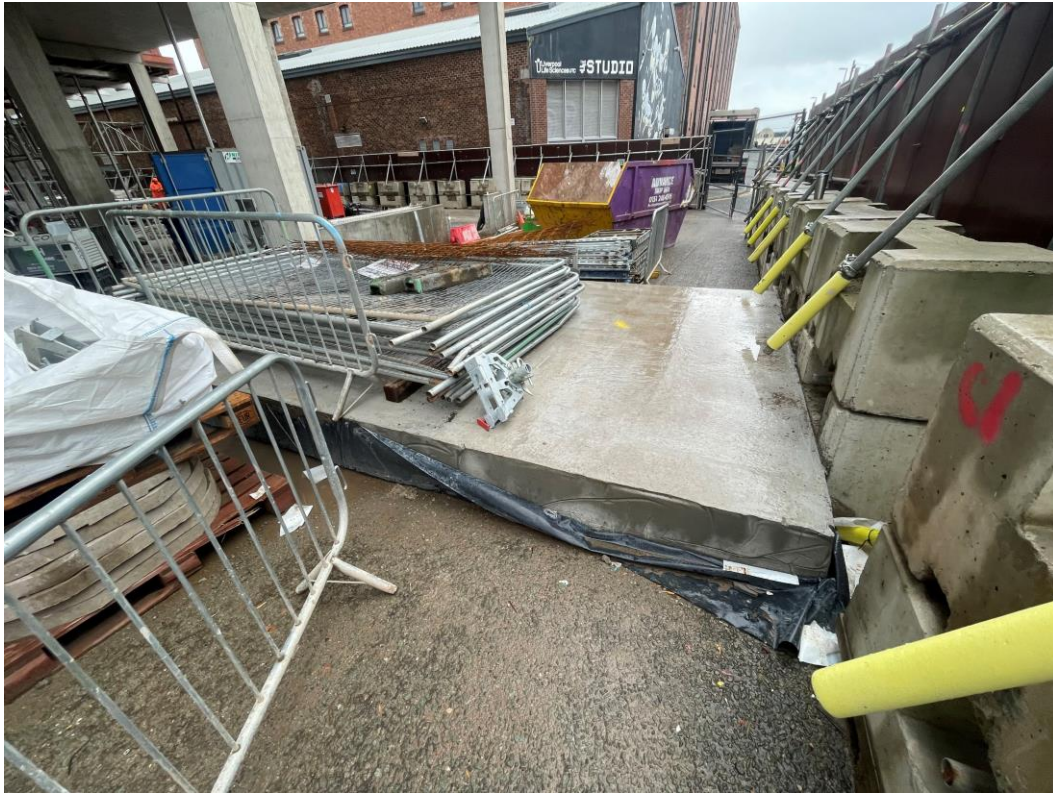
Concrete base poured for Hoist
