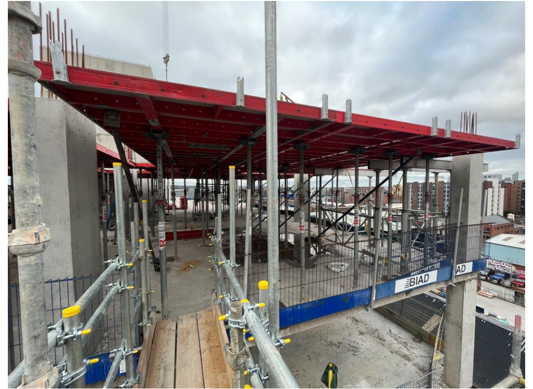
Section A – Formwork in place in preparation for Level 7
