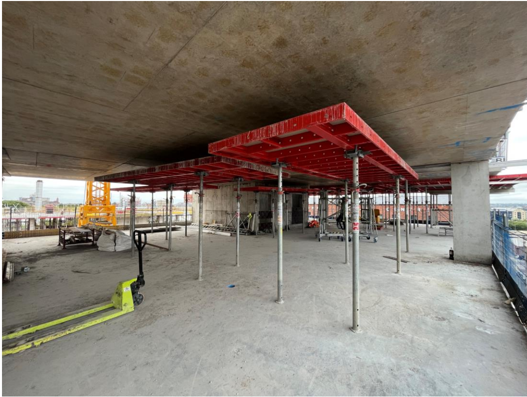
Section B – Removal of form work following Level 5
