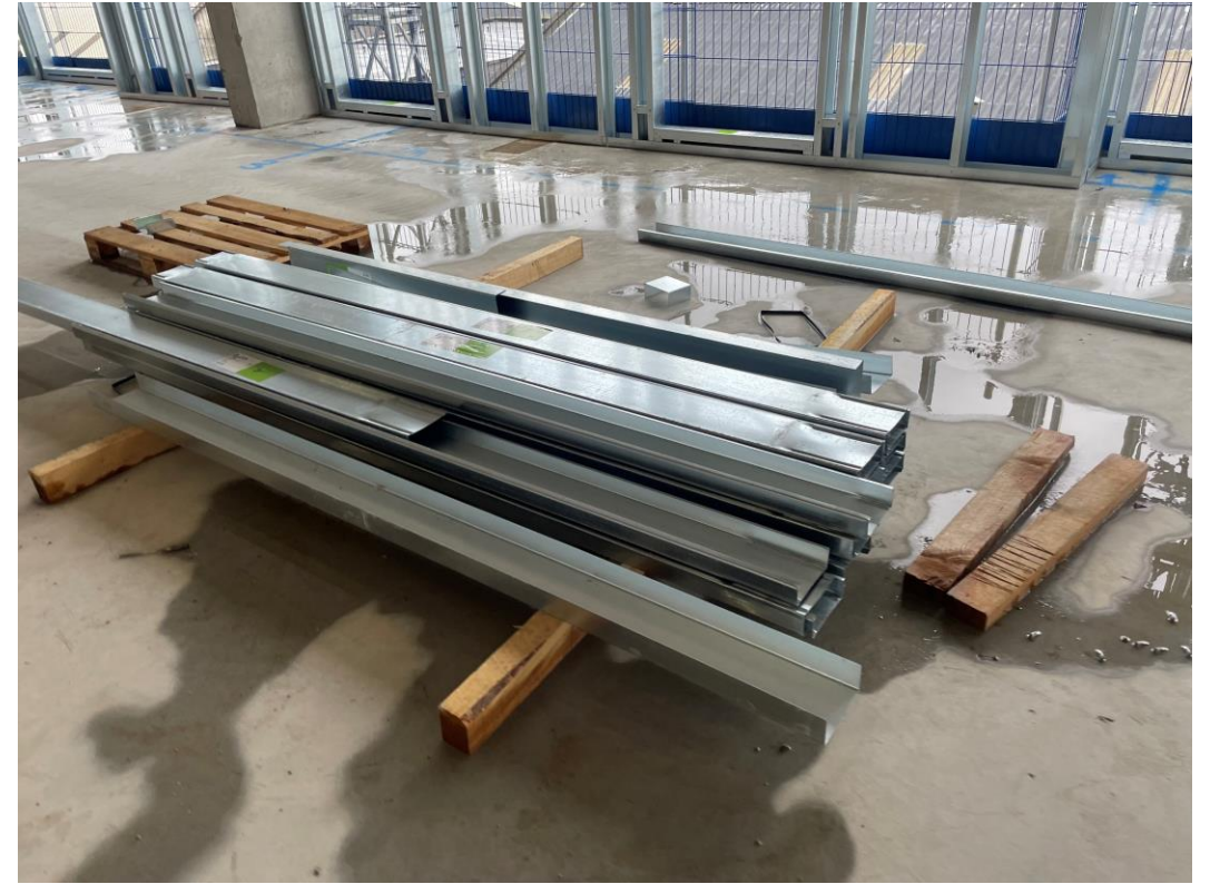
Section A – SFS loaded to Level 2 ready for installation
