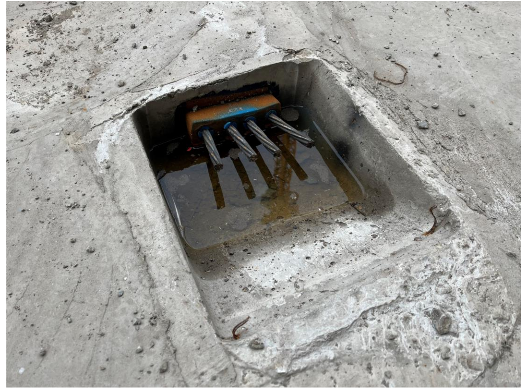
Section C – Installation of PT Strands
