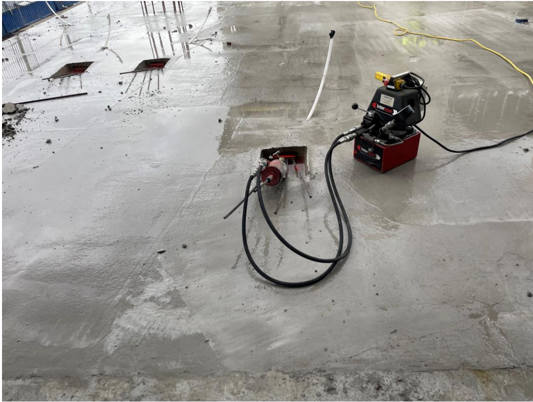
Section C – Installation of PT Strands
