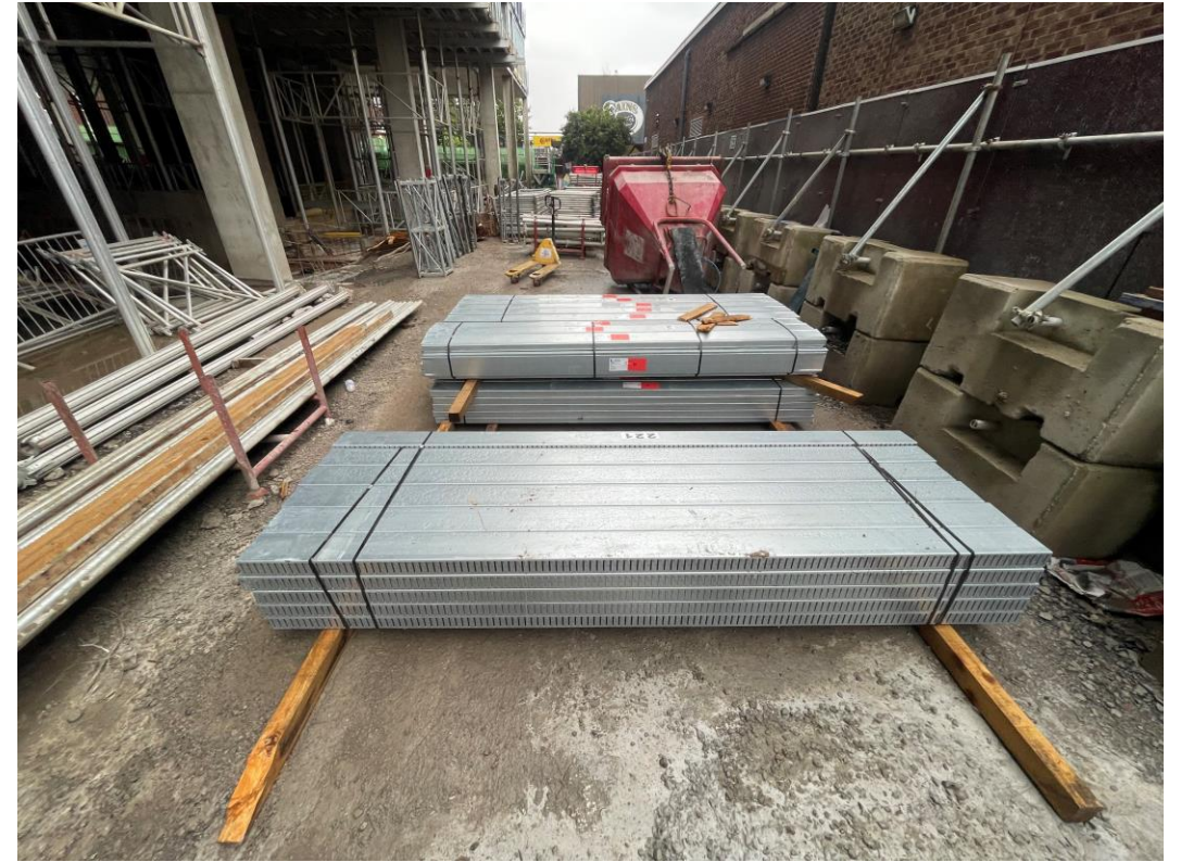
SFS onsite for installation
