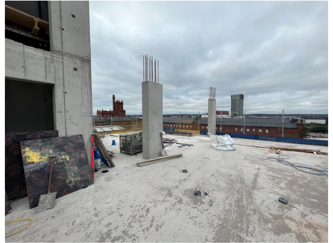
Section A – Concrete frame construction ongoing
