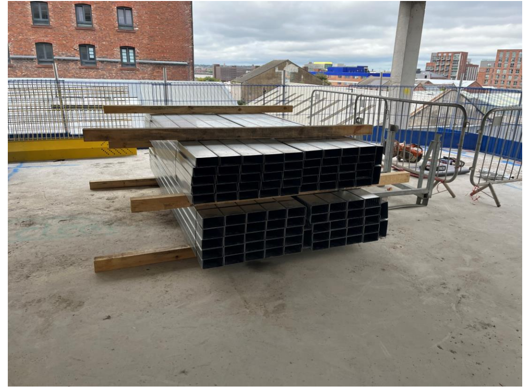
SFS loaded for installation
