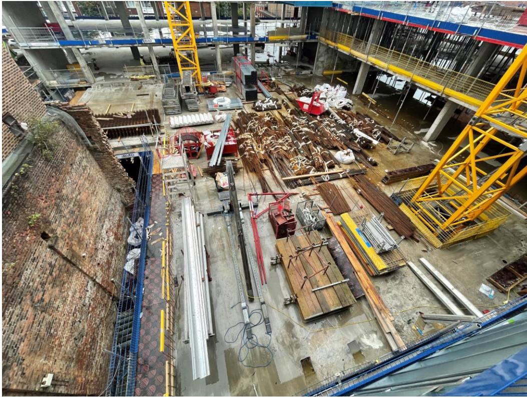
Reinforcement onsite ready for installation
