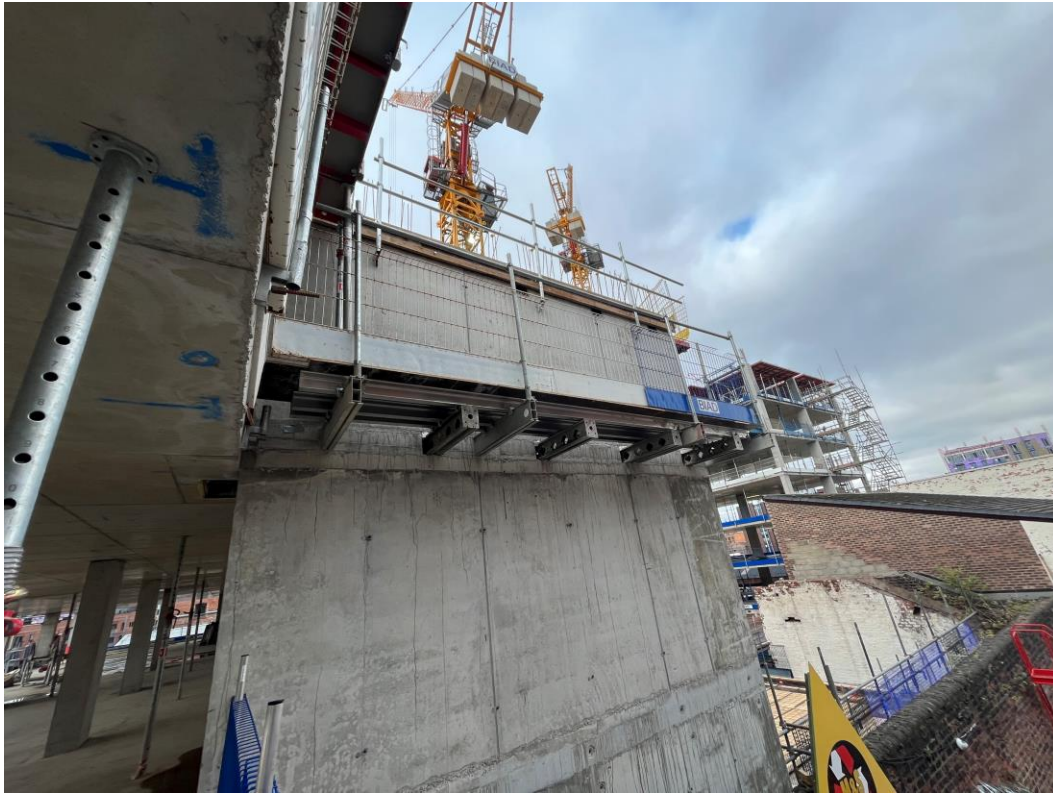
Section B – Temporary working platform in place
