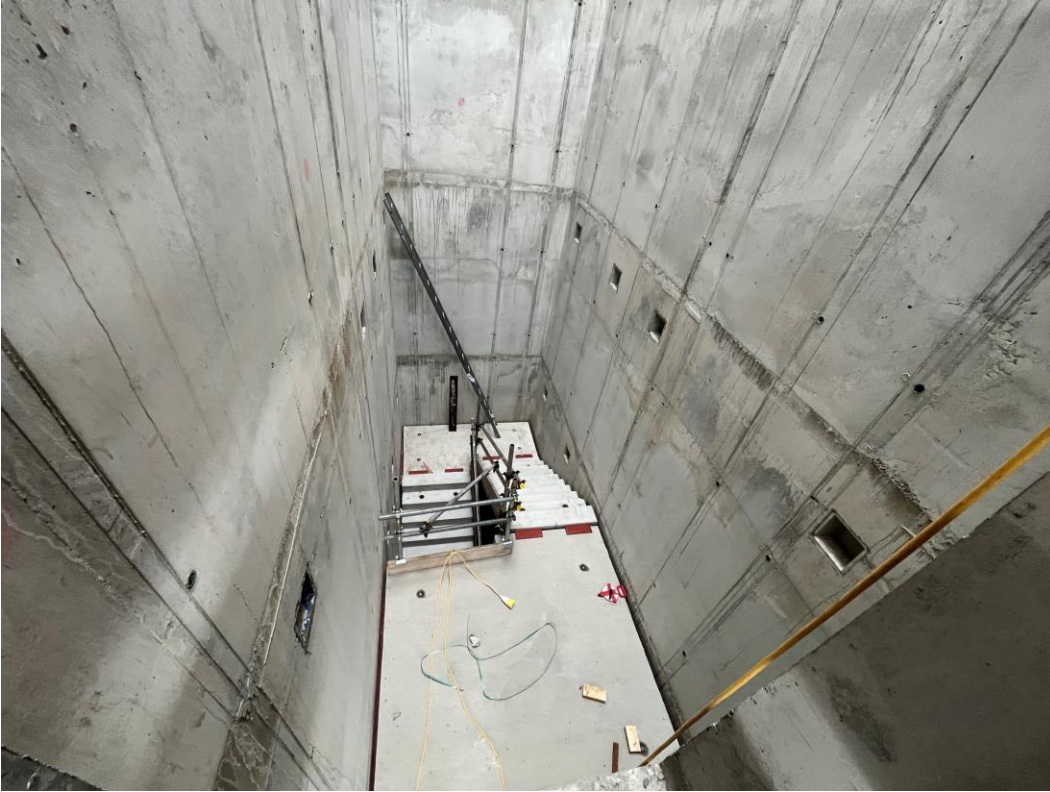
Section A – Concrete stair case installation ongoing
