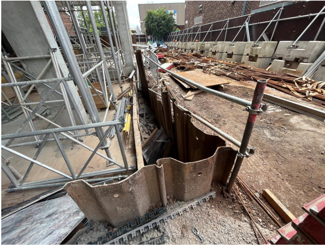
Section A – Sheet piling in place
