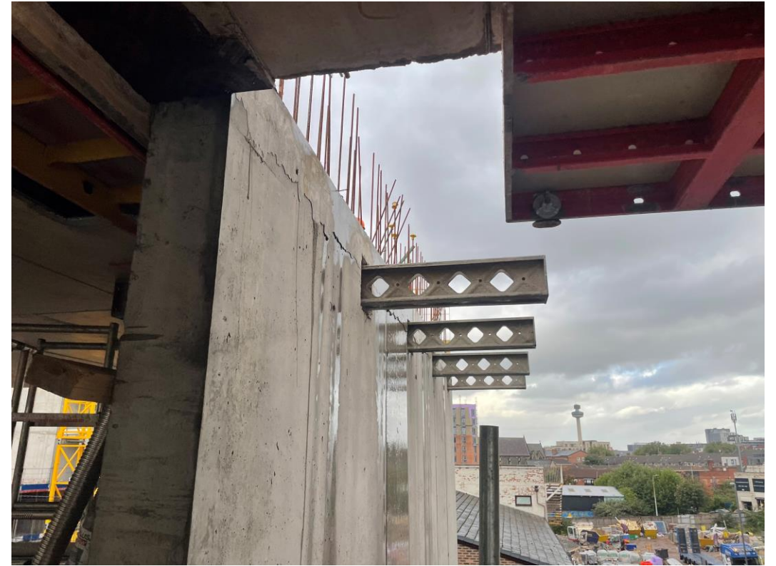
Section B – Formwork support in place
