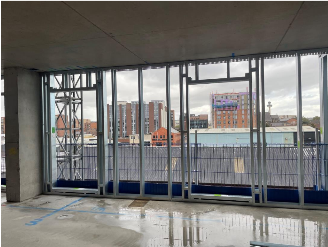
Section A – SFS Installation commenced
