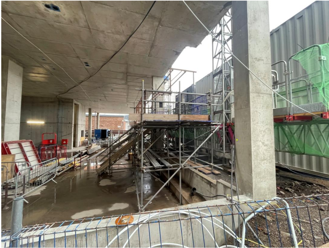
Section A – Mast Climber access in place
