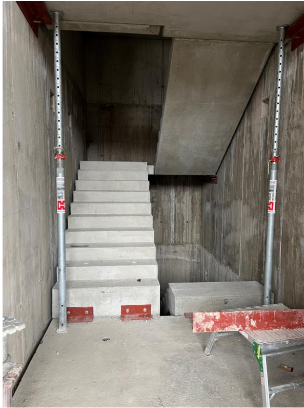
Stair Core 1 - Concrete stair installation has commenced
