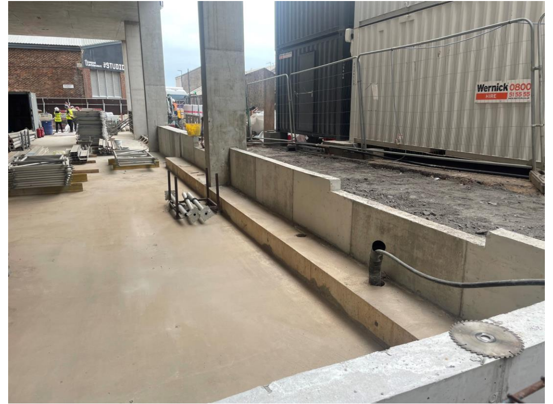
Section A – Concrete upstand
