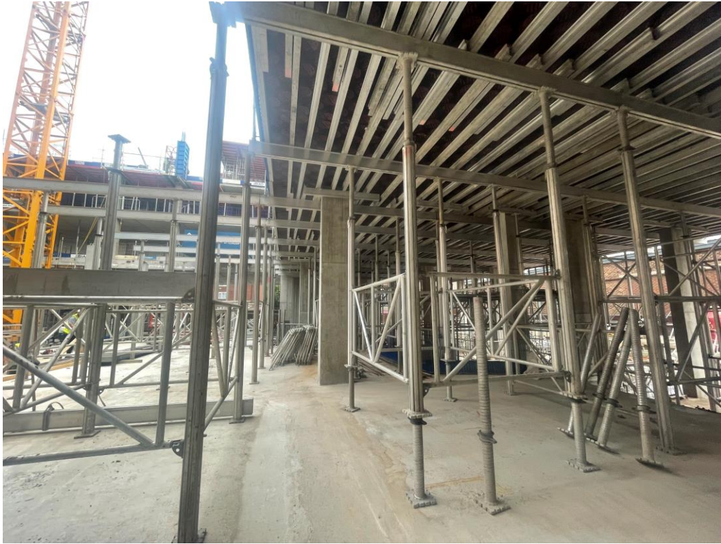
Section C – Formwork supports
