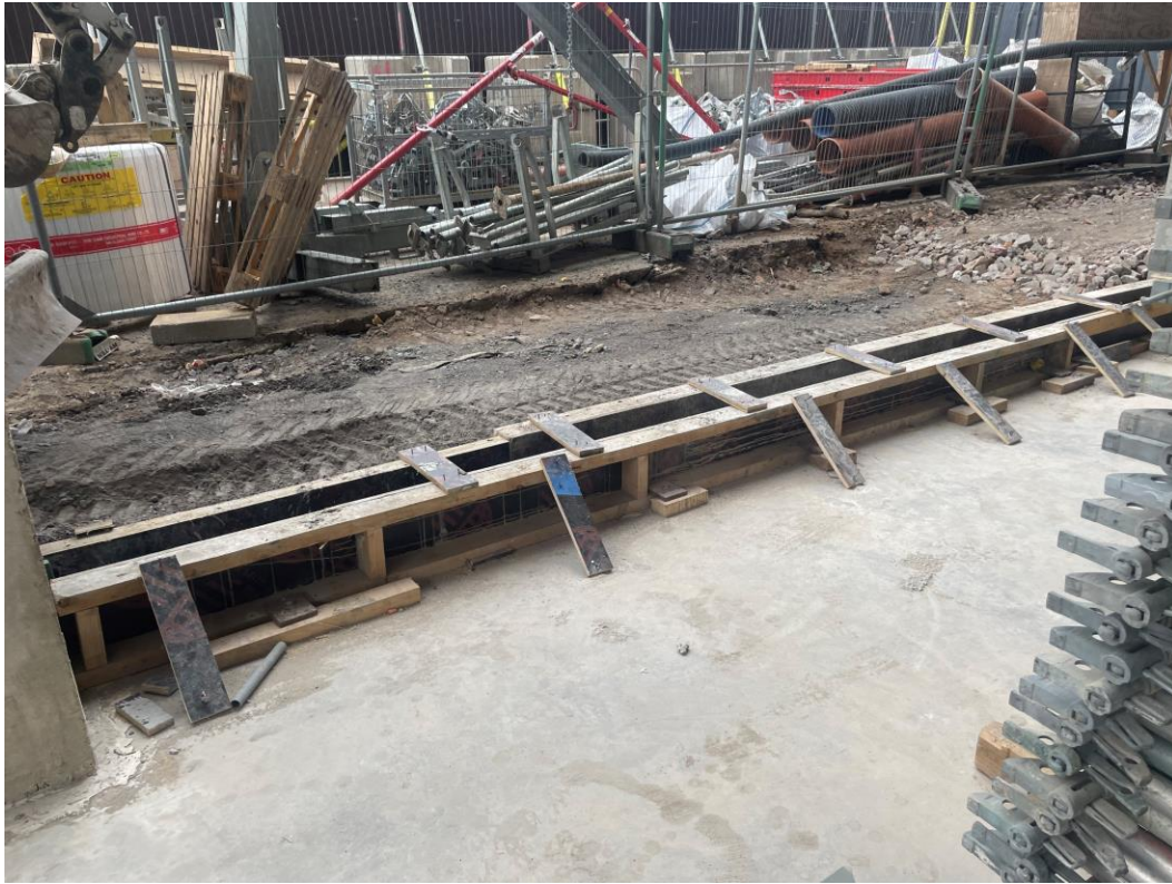
Section A - Formwork for concrete upstand
