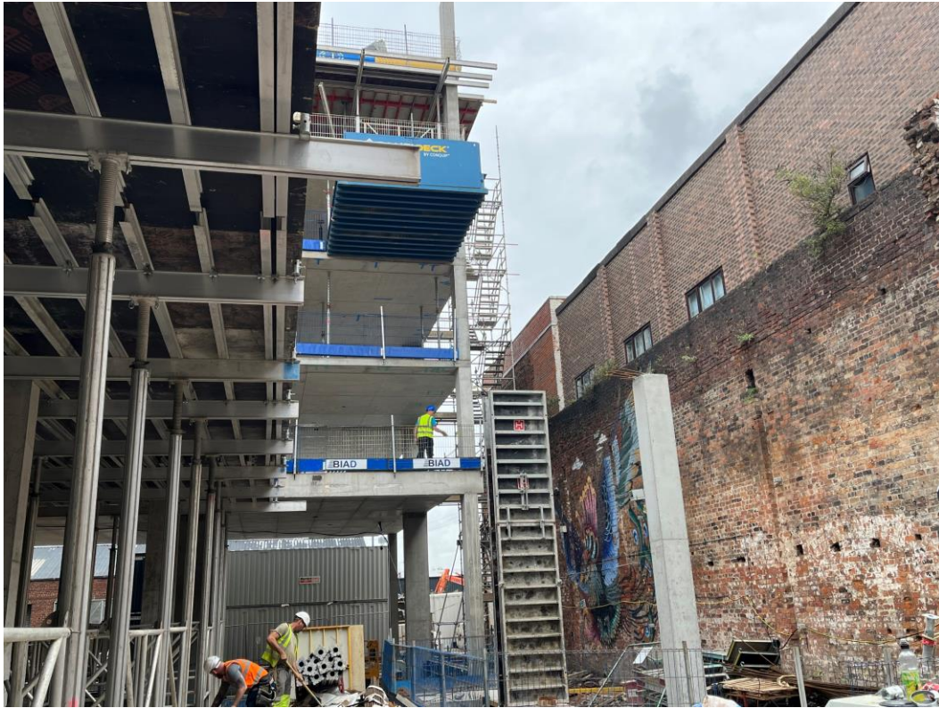
Section A – Reinforced frame construction ongoing
