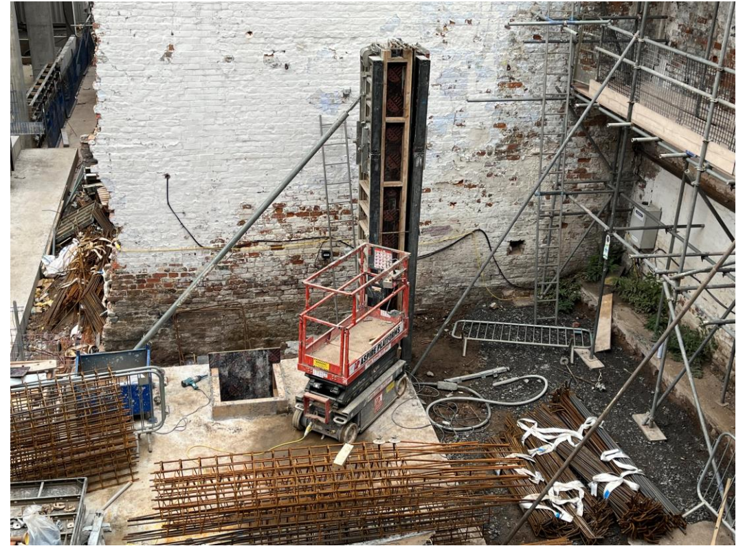
Podium - Columns & slab formwork in place.
