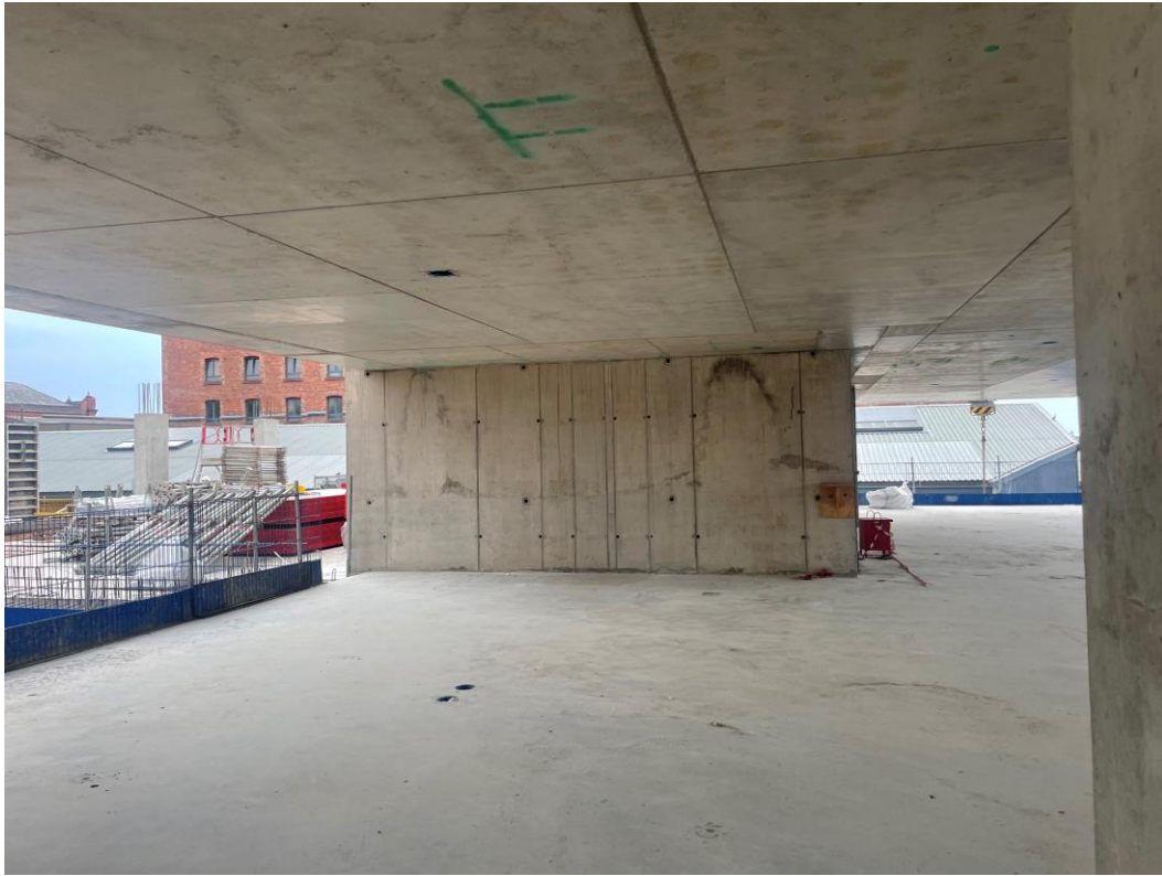
Section A – Level 2 formwork supports removed following slab pour
