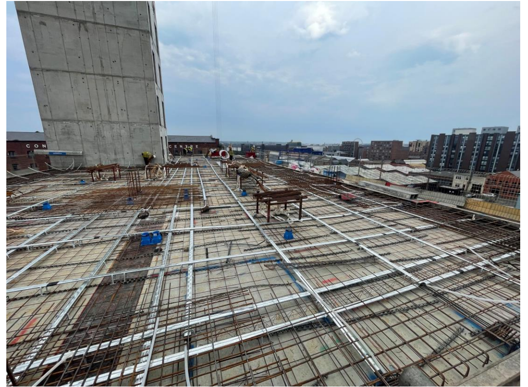
Section A – Reinforcement laid in preparation for Level 5 slab pour
