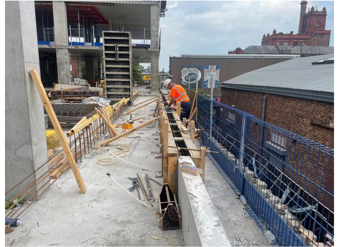
Section C - Formwork for concrete upstand
