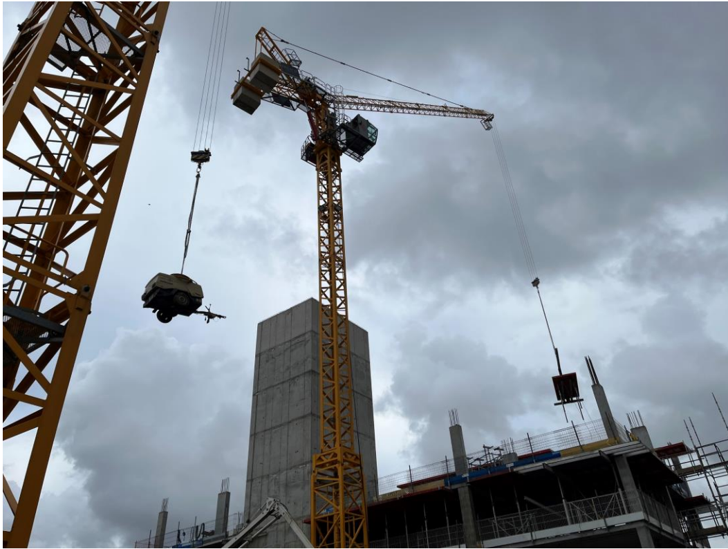
Cranes in operation
