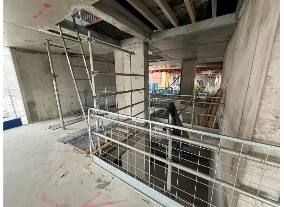
Section B – Reinforced frame construction ongoing
