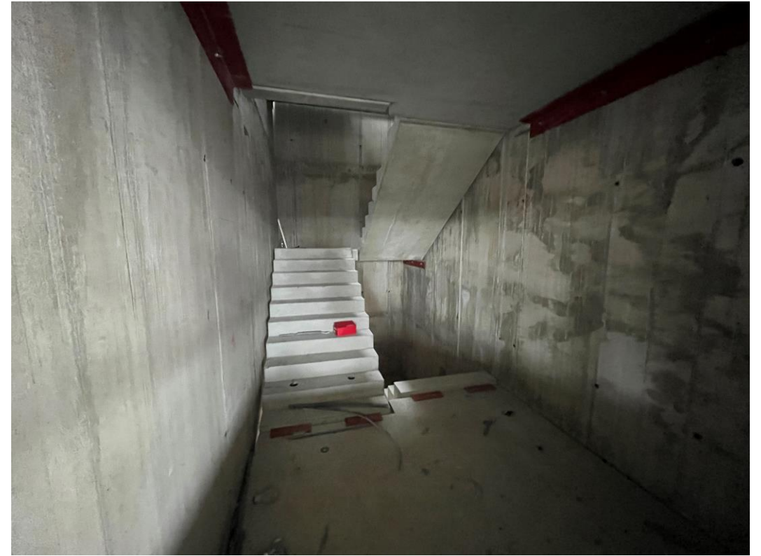
Stair Core 1 - Concrete stair installation has commenced
