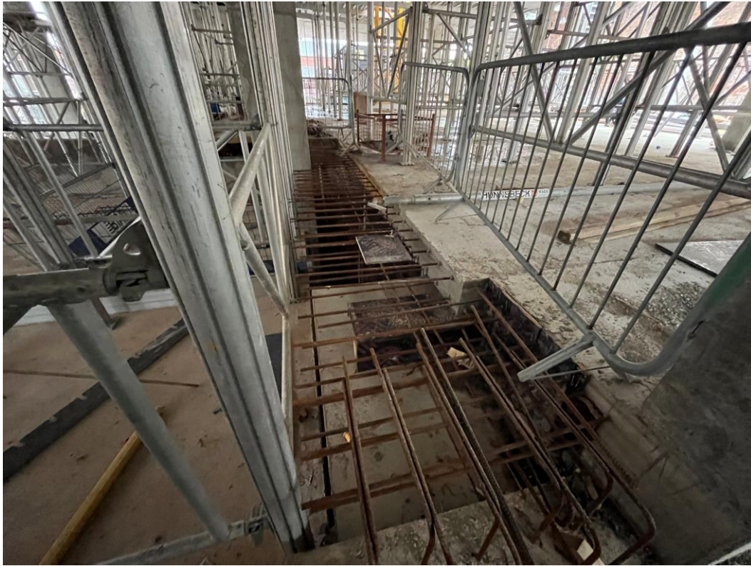
Section C – Reinforced frame construction ongoing
