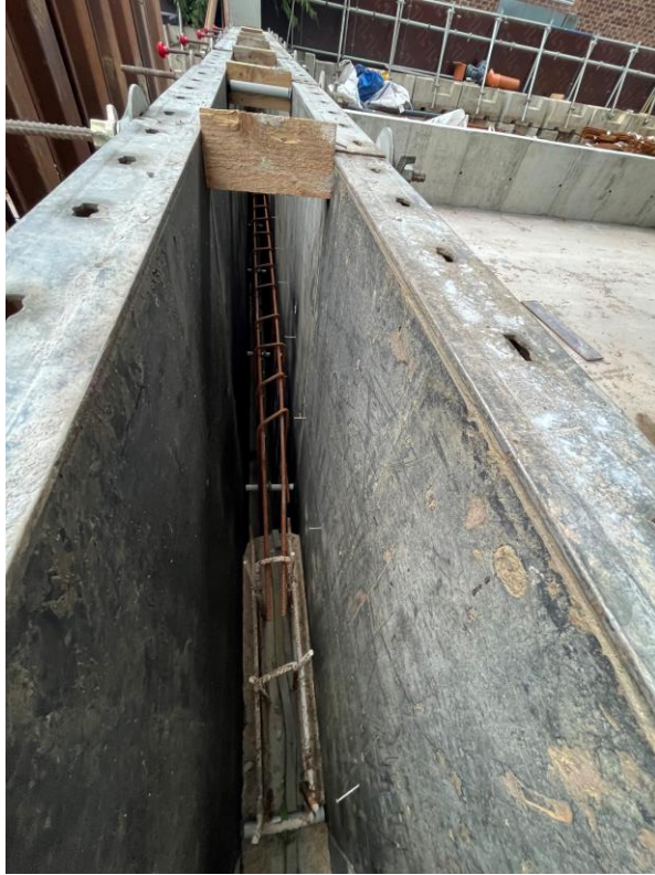
Formwork for retaining wall casting in place
