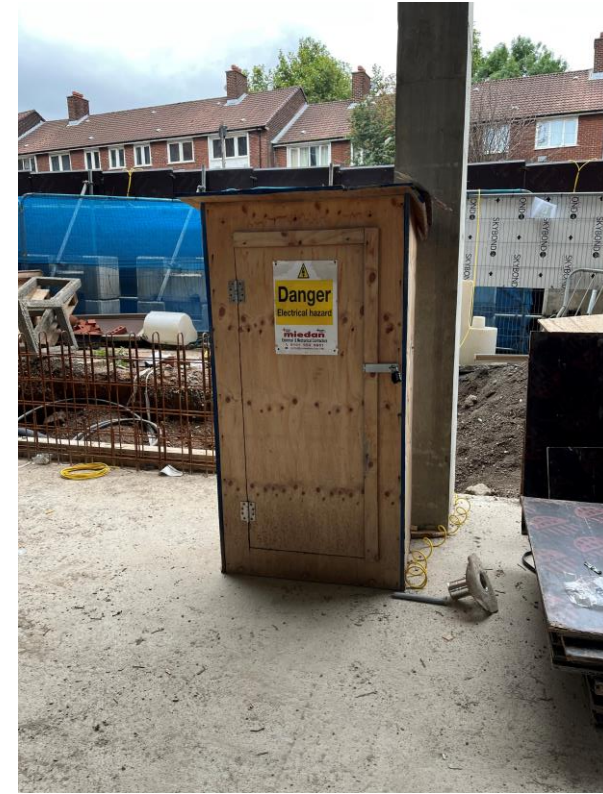
Section A – Temporary electrical supply installed
