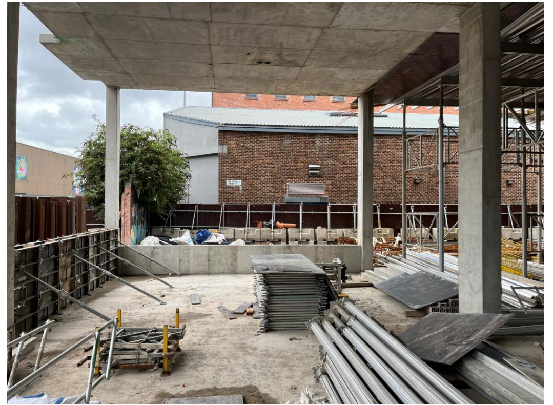
Section B – Reinforced frame construction ongoing
