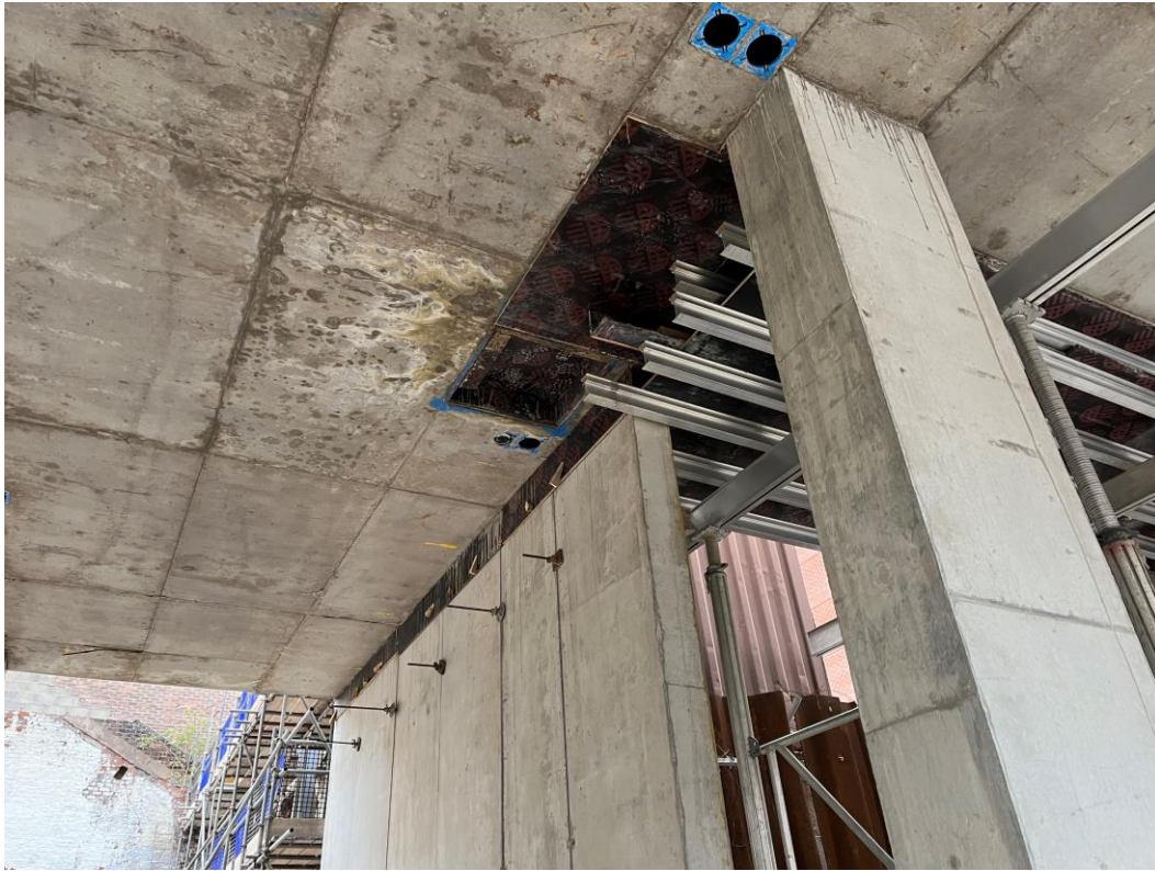
Section A – Reinforced frame construction ongoing
