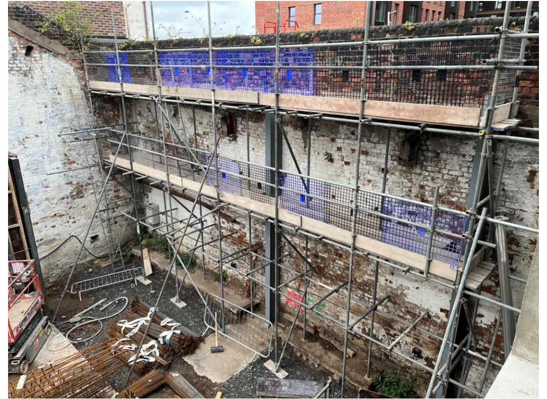
Party wall steel support works ongoing
