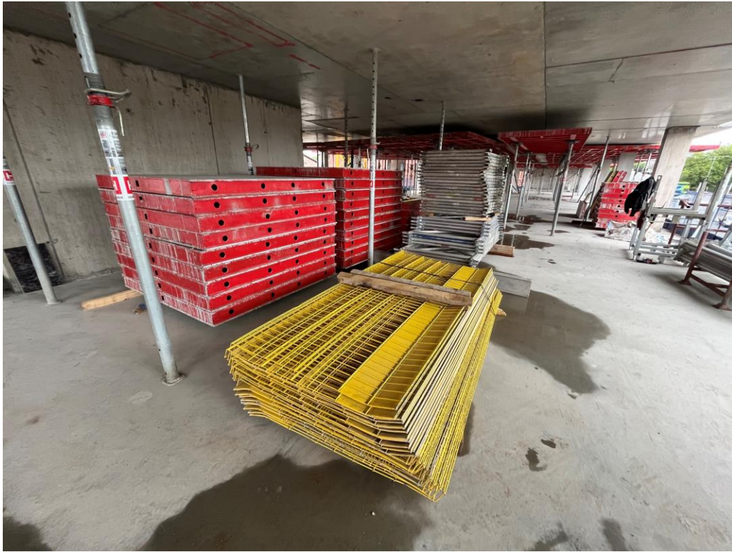
Floor slab formwork onsite
