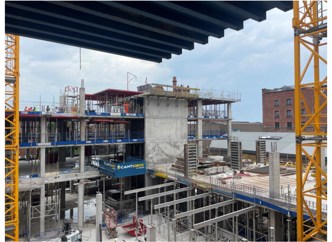
Section B – Level 4 slab formwork installation has commenced
