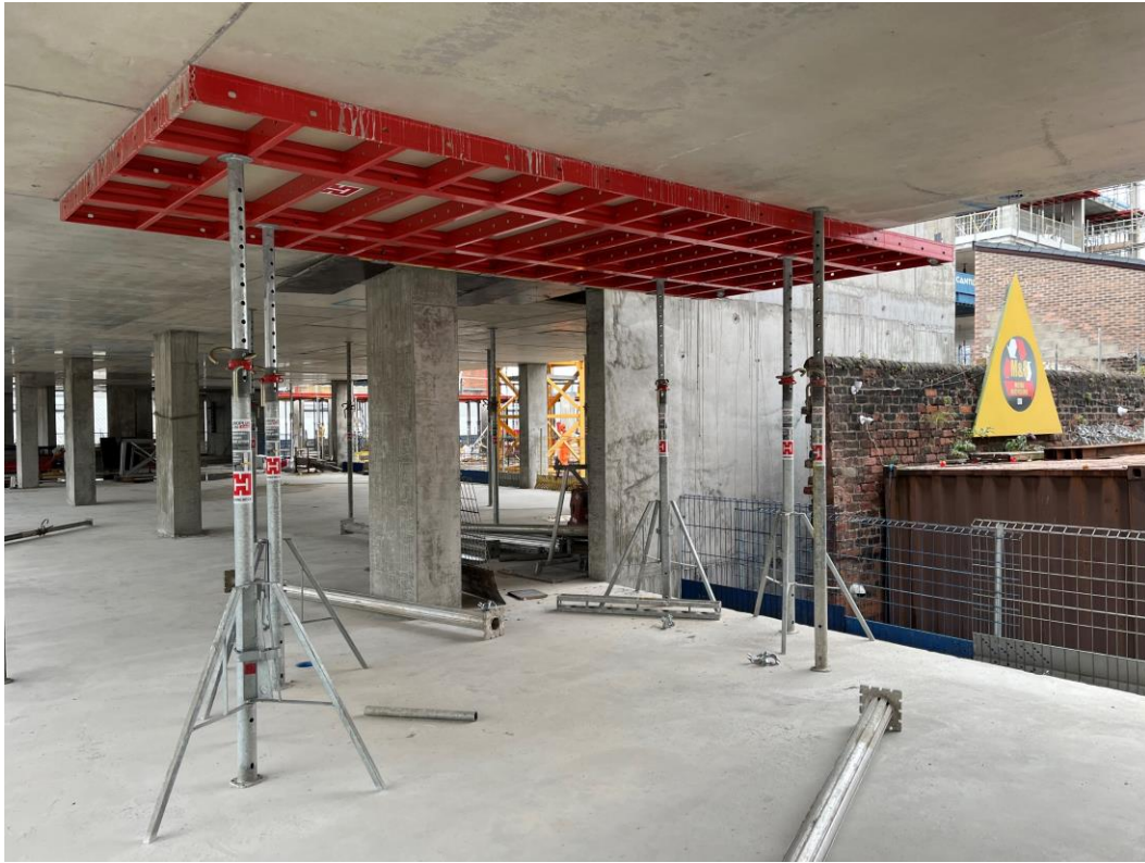
Section C – Formwork in place for Level 1 slab pour
