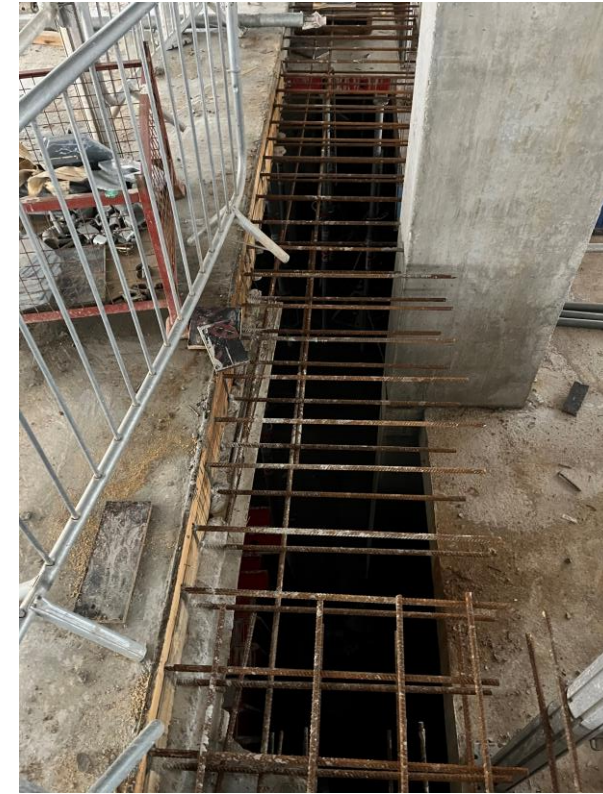
Section A – Reinforced frame construction ongoing
