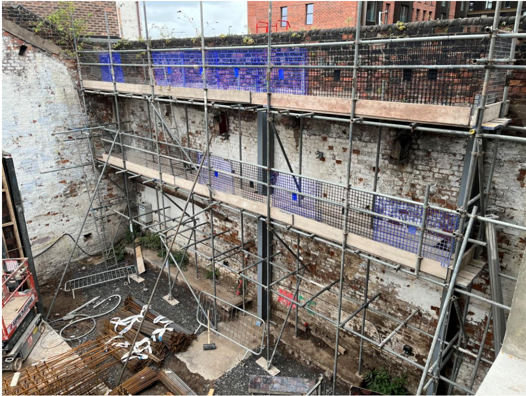
Party wall works
