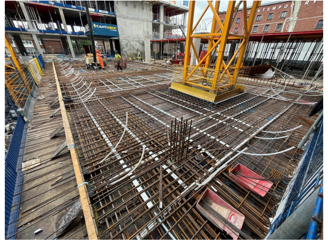
Podium – Reinforcement laid in preparation for slab pour
