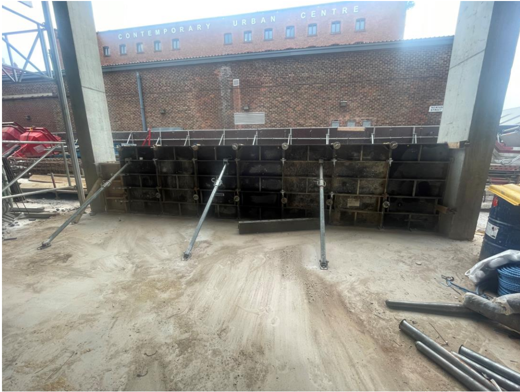
Section A – Formwork in place for retaining wall
