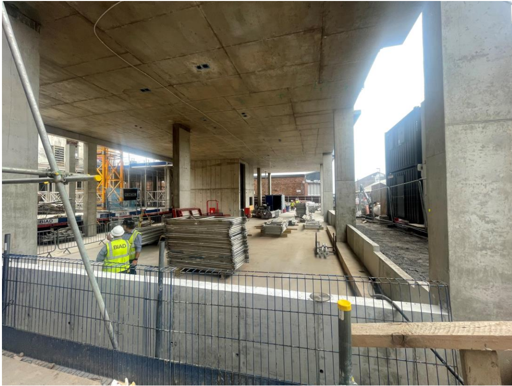
Section A – Formwork removed
