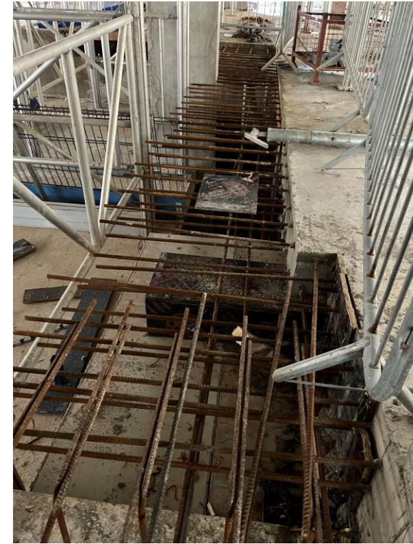
Section C – Reinforced frame construction ongoing
