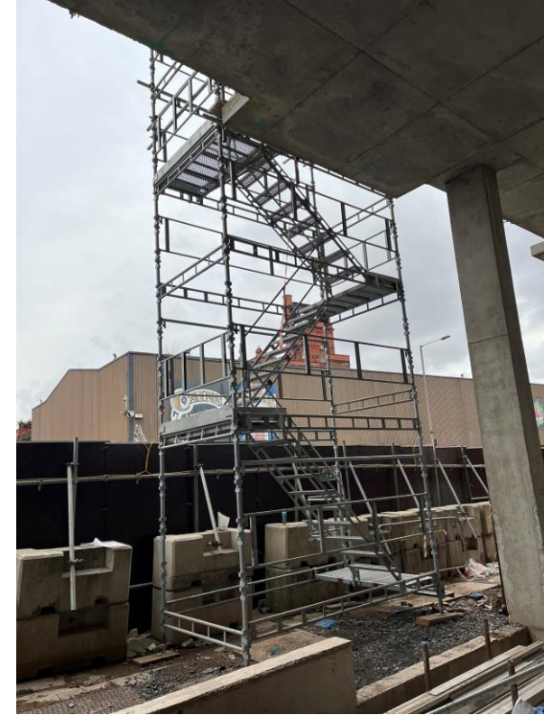
Section B – Haki staircase installed
