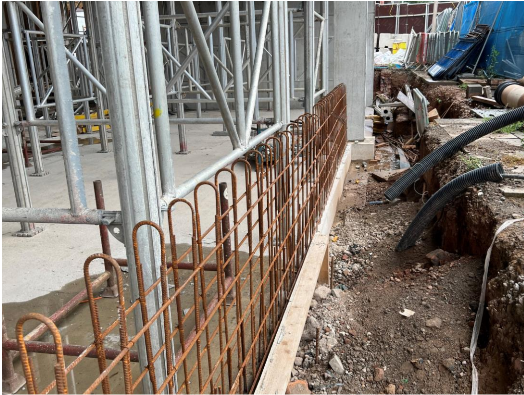
Reinforcement for concrete upstand
