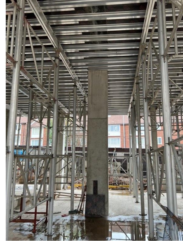
Formwork for slab casting in place
