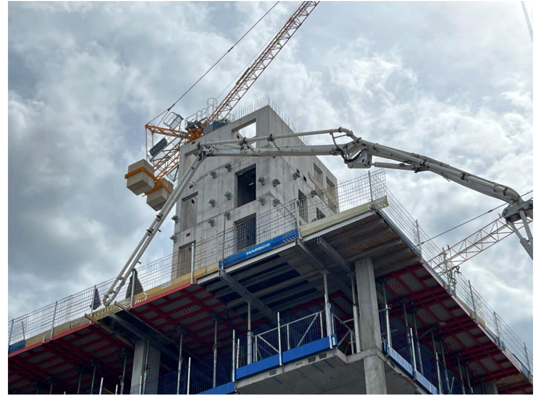
Zone A – Stair core construction complete
