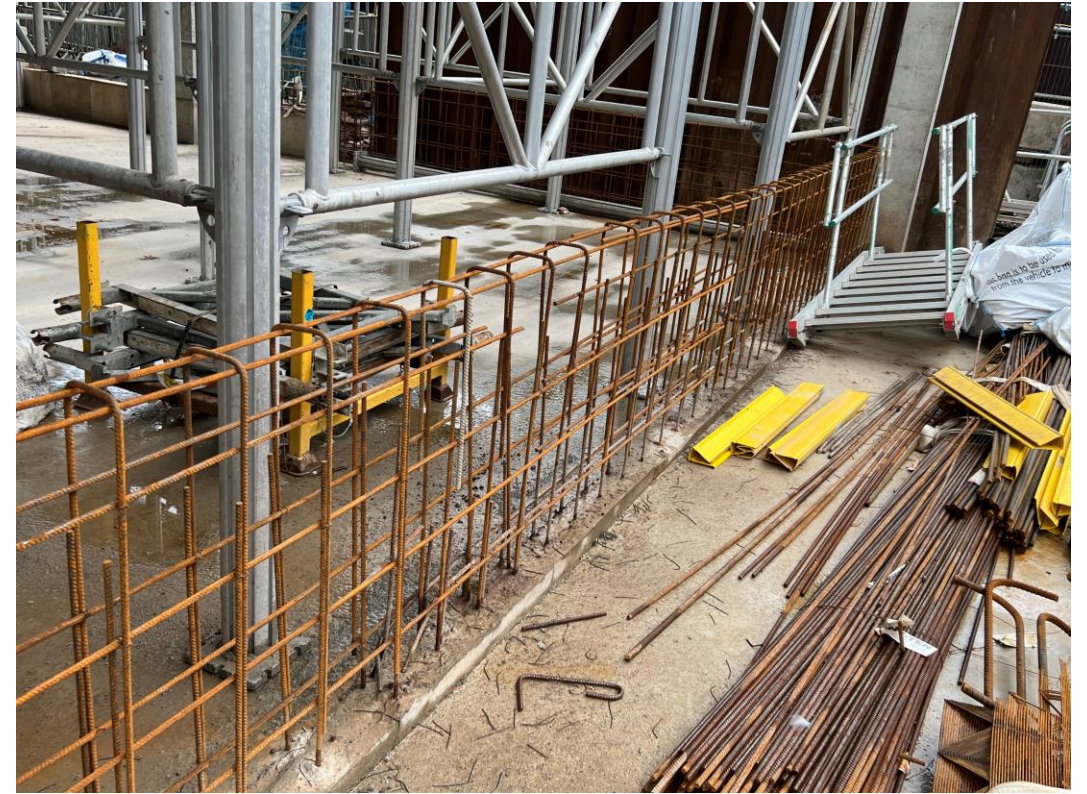
Reinforcement for concrete upstand
