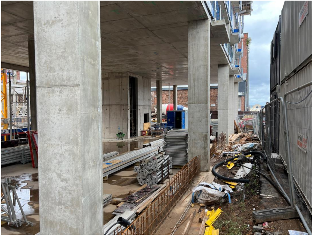
Zone A – Reinforced frame construction
