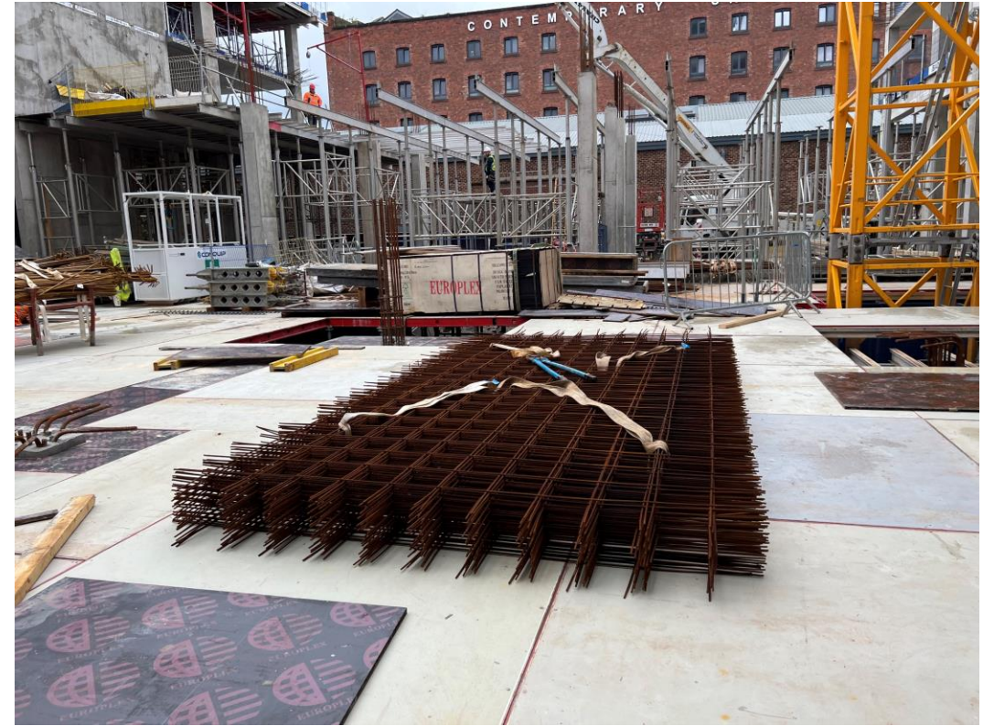
Zone C – Concrete reinforcement onsite for installation
