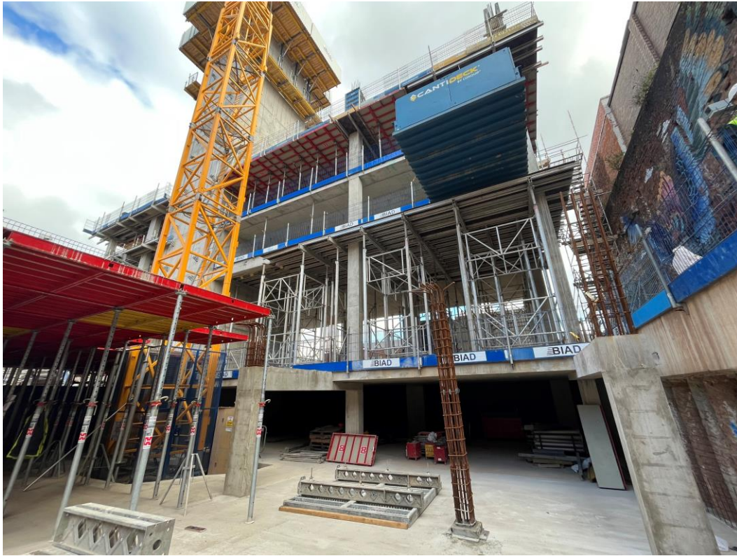
Zone A – Formwork for upper floor slabs installed
