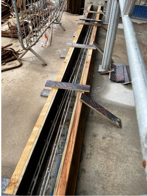
Shuttering in place for retaining wall concrete pour
