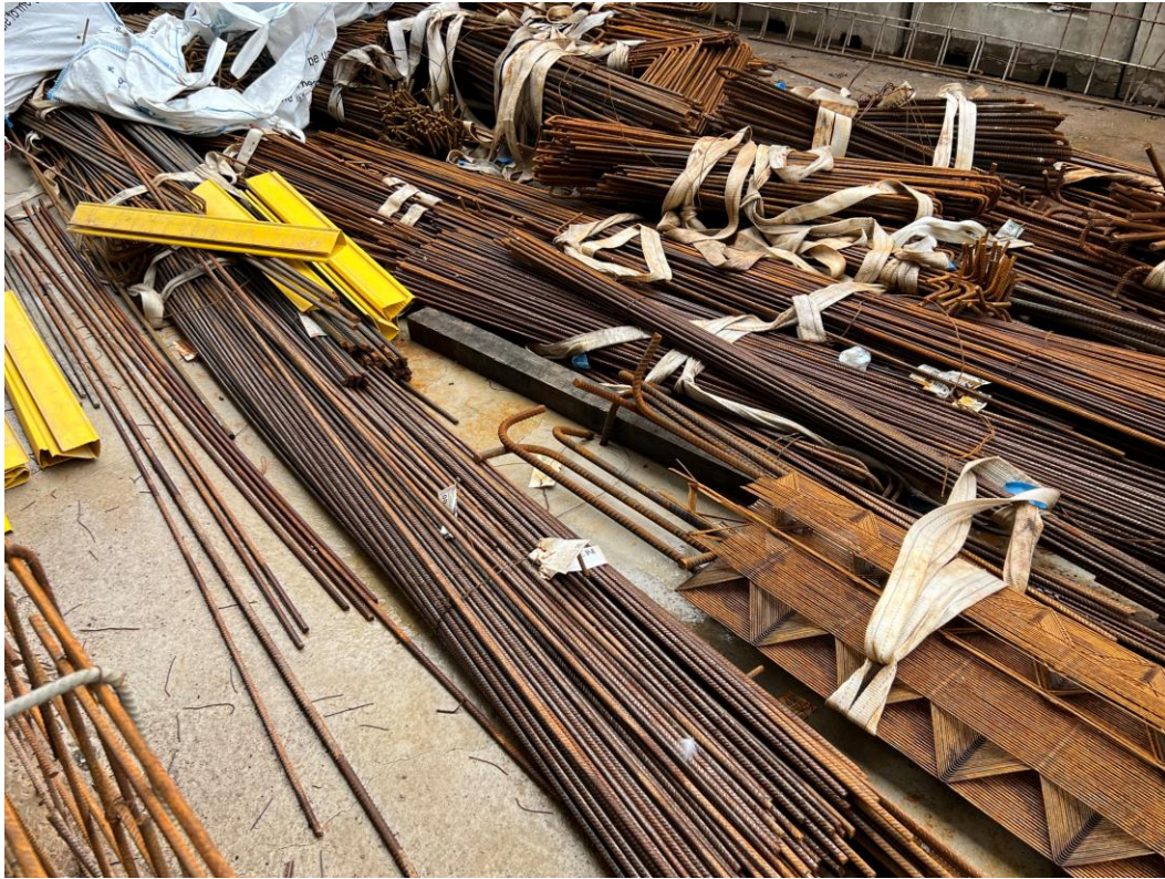
Reinforcement onsite for installation
