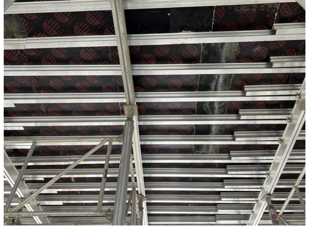
Formwork for slab casting in place
