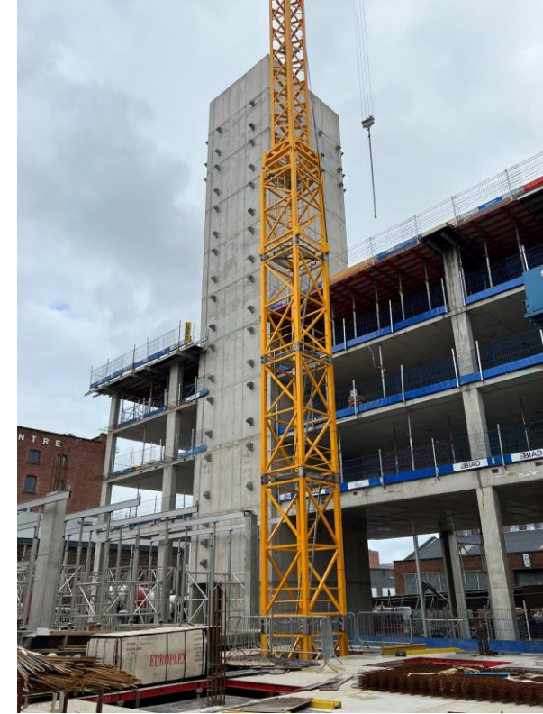
Zone A – Reinforced frame construction ongoing
