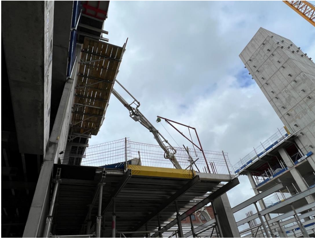
Zone A – Reinforced concrete frame construction ongoing
