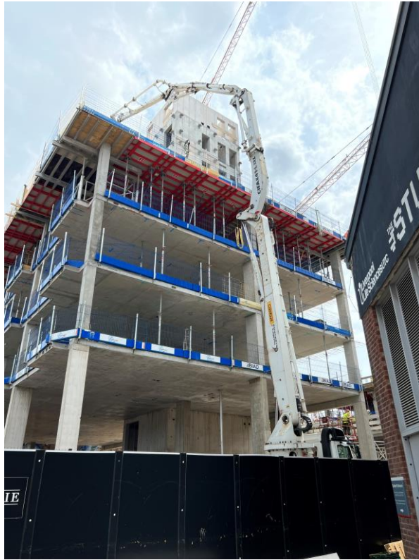
Block D – Reinforced concrete frame construction ongoing
