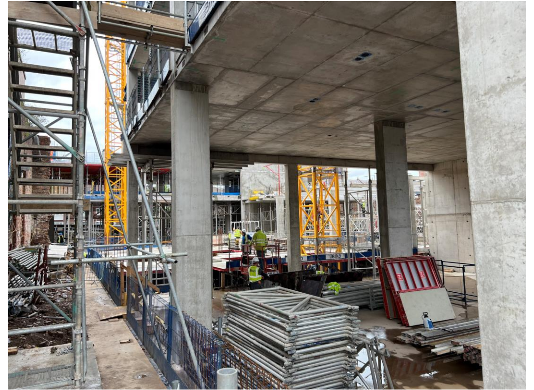
Zone A – Reinforced frame construction
