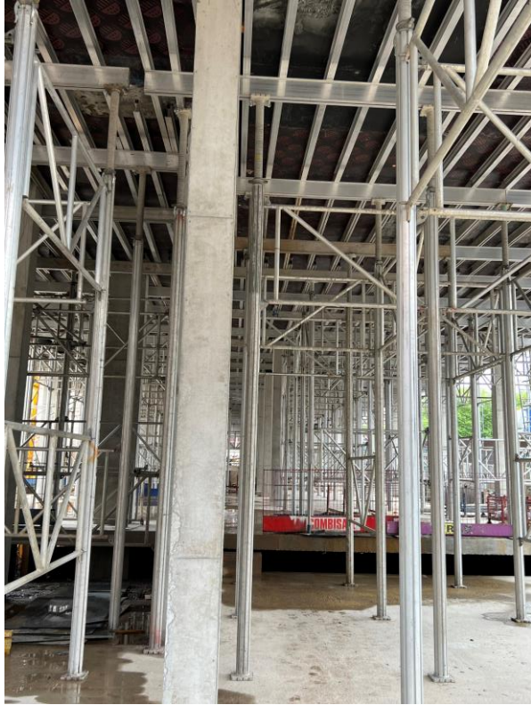
Formwork for upper floor slabs installed
