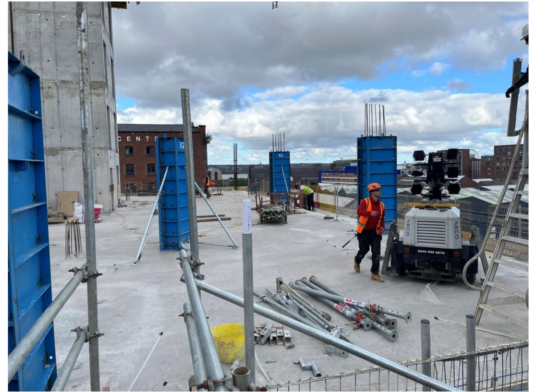
Zone B – 2nd Floor slab cast
