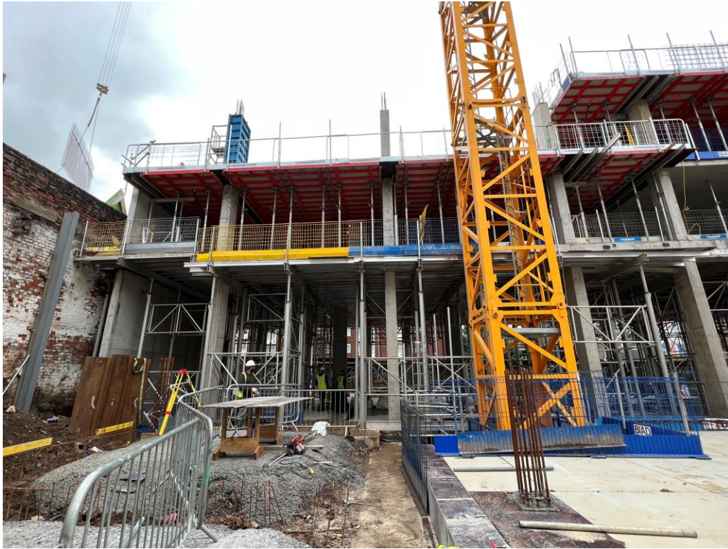
Zone A – Reinforced frame construction ongoing
