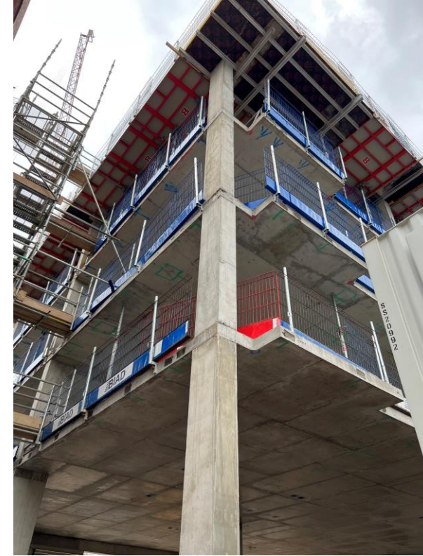
Zone A – Reinforced concrete frame construction ongoing
