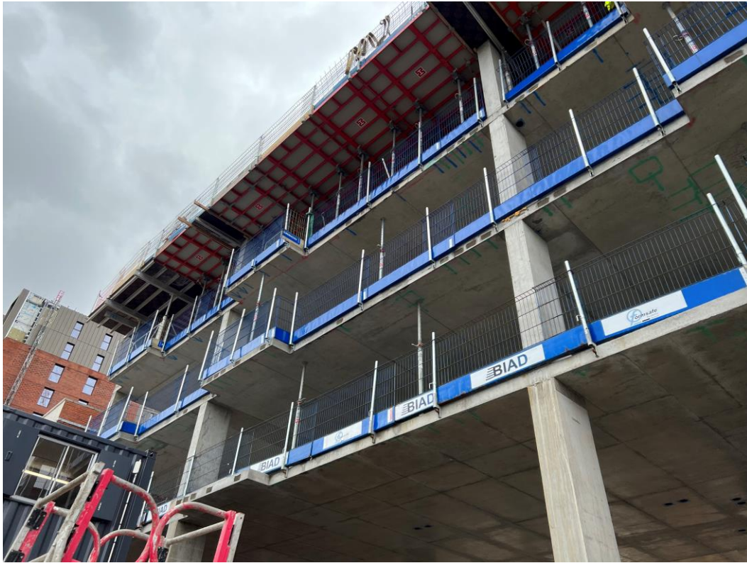
Zone A – Reinforced frame construction ongoing
