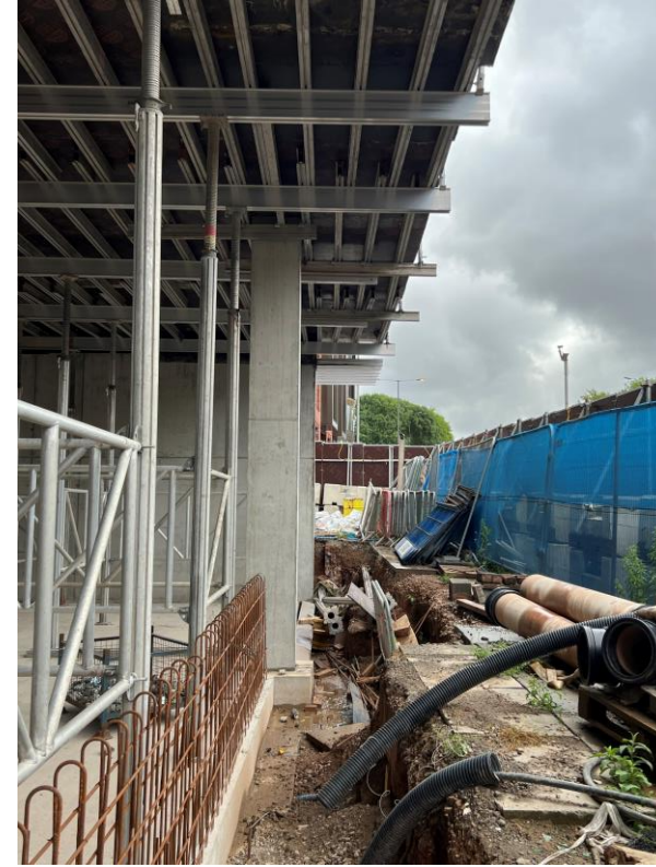
Zone A – Reinforced frame construction
