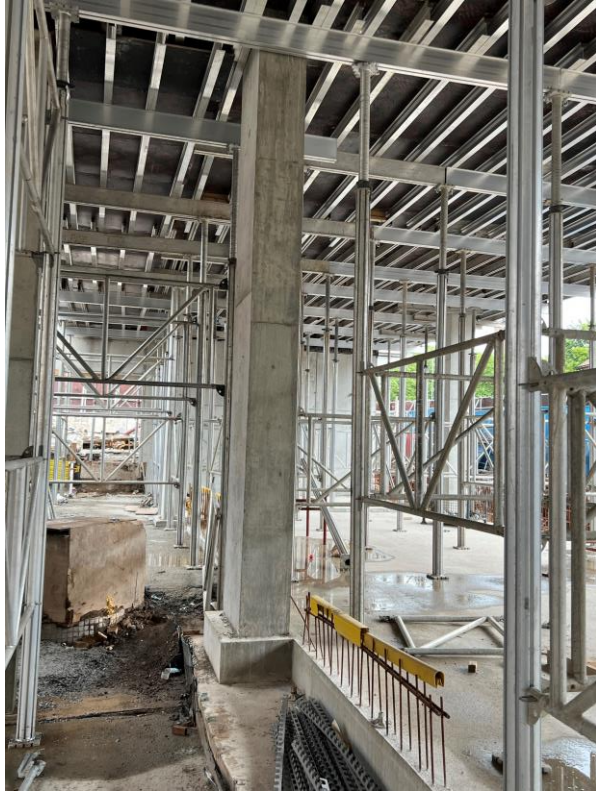
Formwork for slab casting in place
