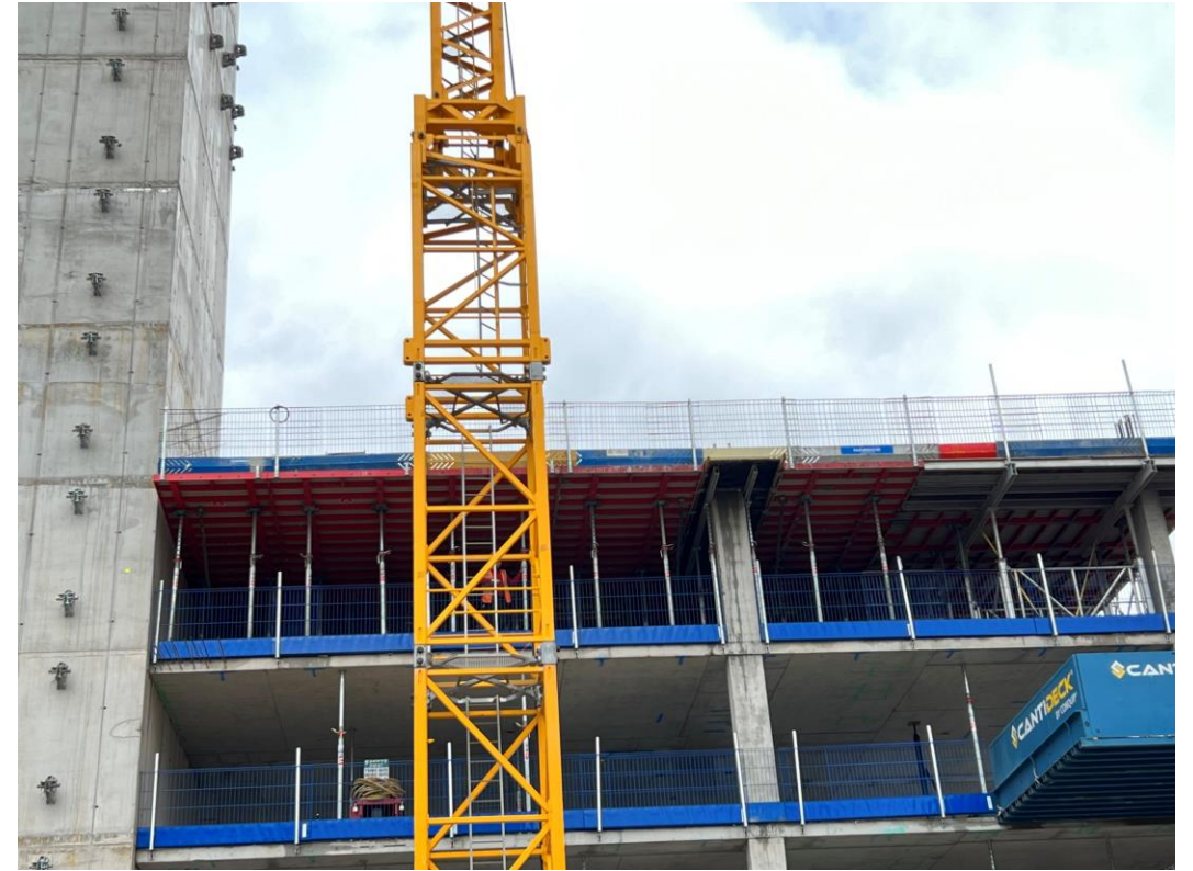
Zone A – reinforced concrete frame construction ongoing
