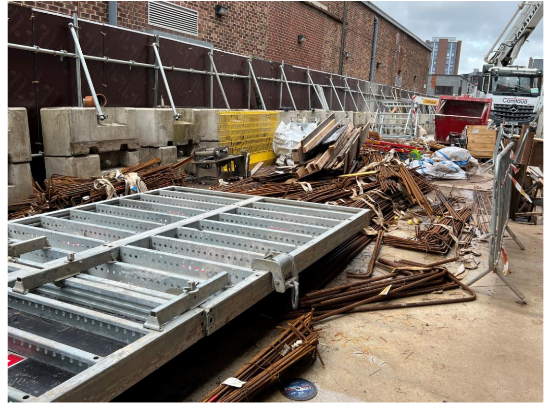
Formwork onsite for casting
