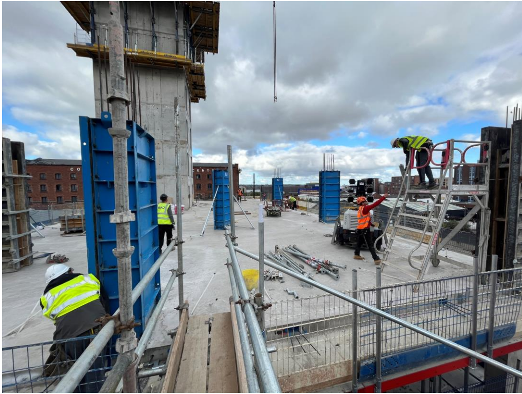
Zone A – 3 rd Floor columns cast
