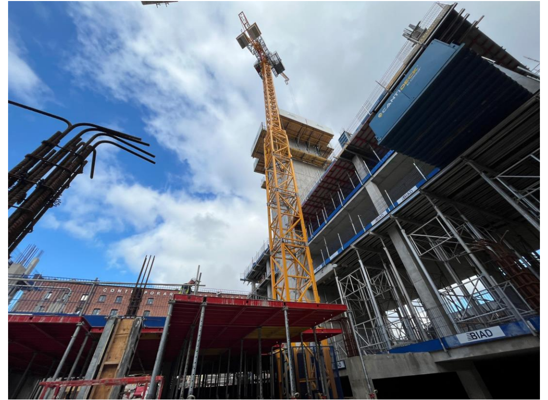
Zone C – Formwork for upper floor slabs installed
