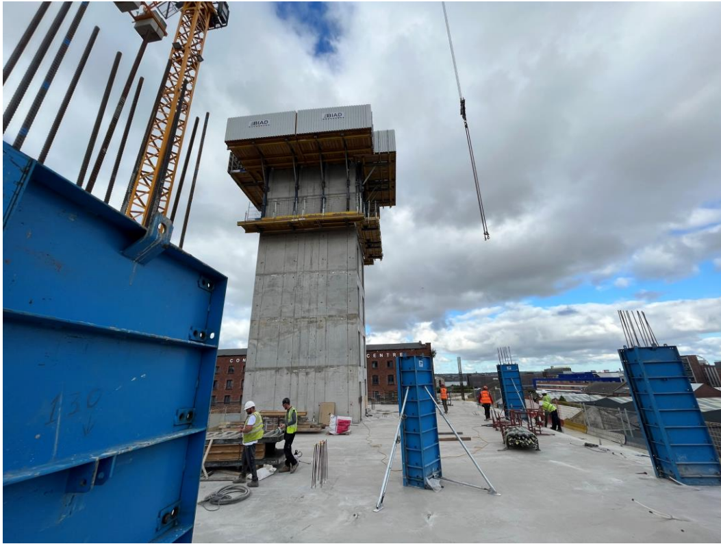
Zone A – Reinforced concrete frame construction ongoing
