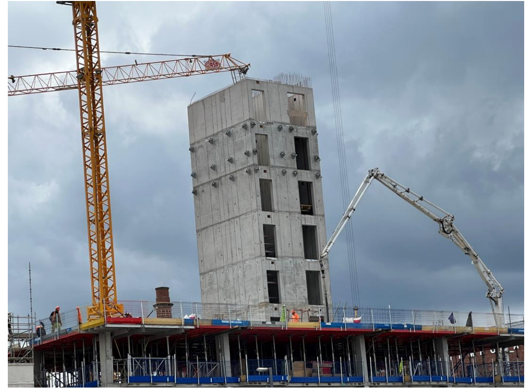
Zone A – Stair core construction complete
