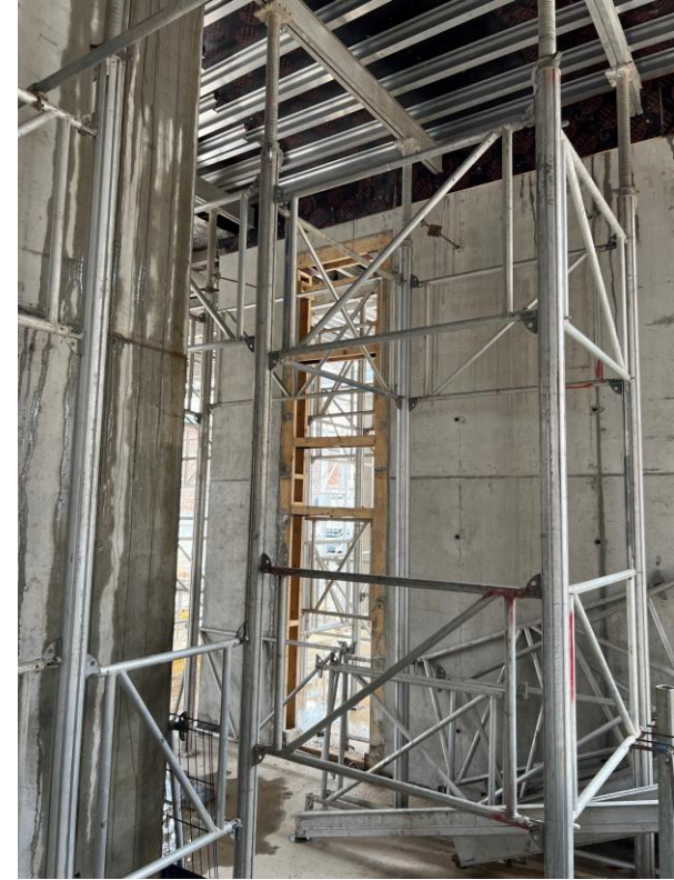
Formwork for upper floor slabs installed
