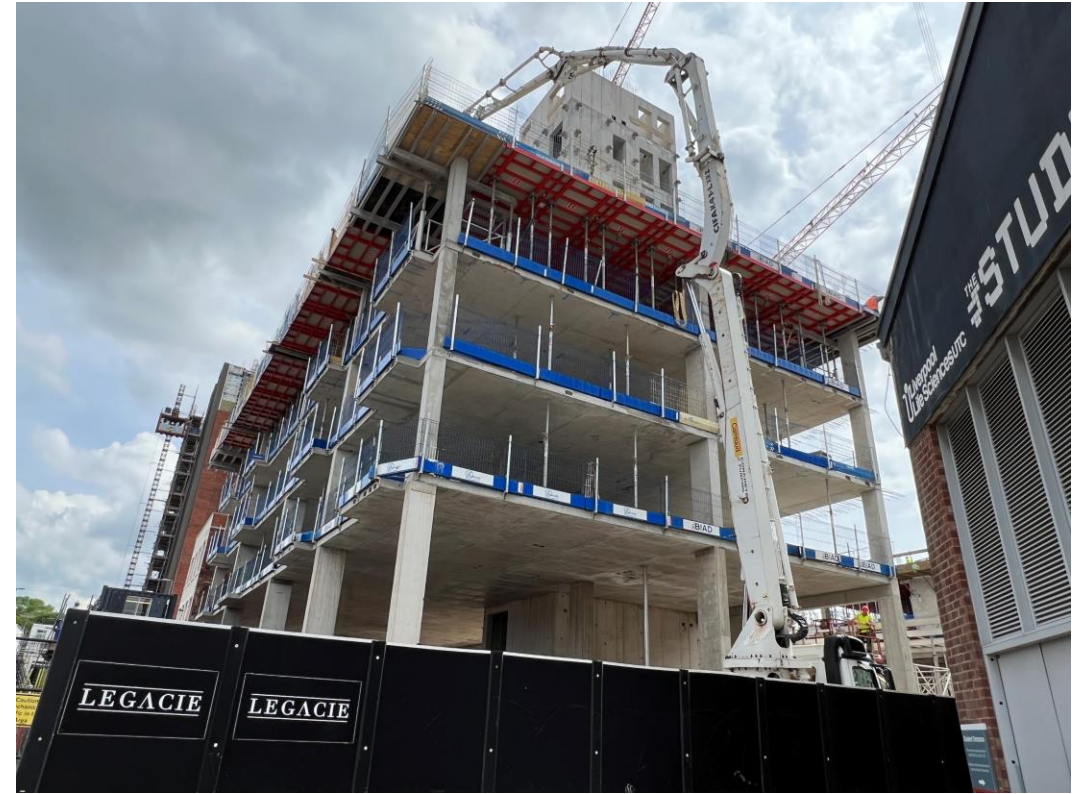
Block D – Reinforced concrete frame construction ongoing
