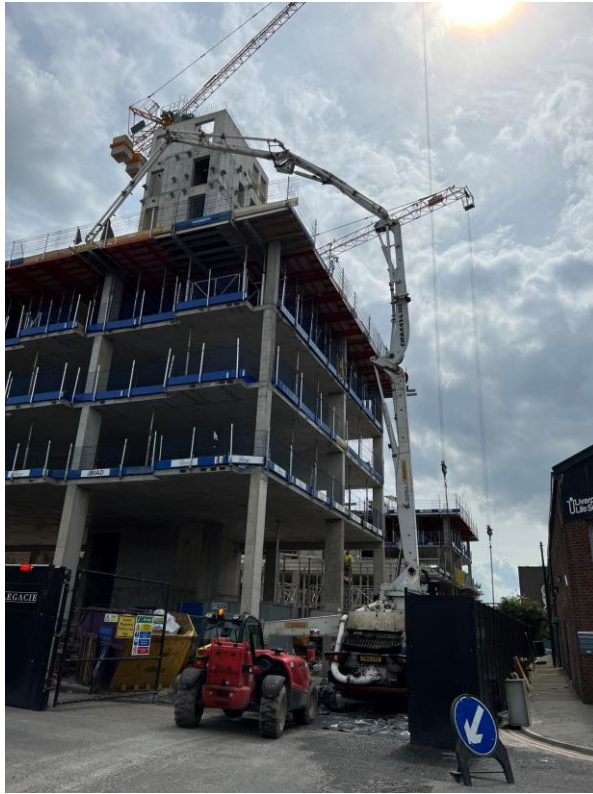
Block D – Reinforced concrete frame construction ongoing
