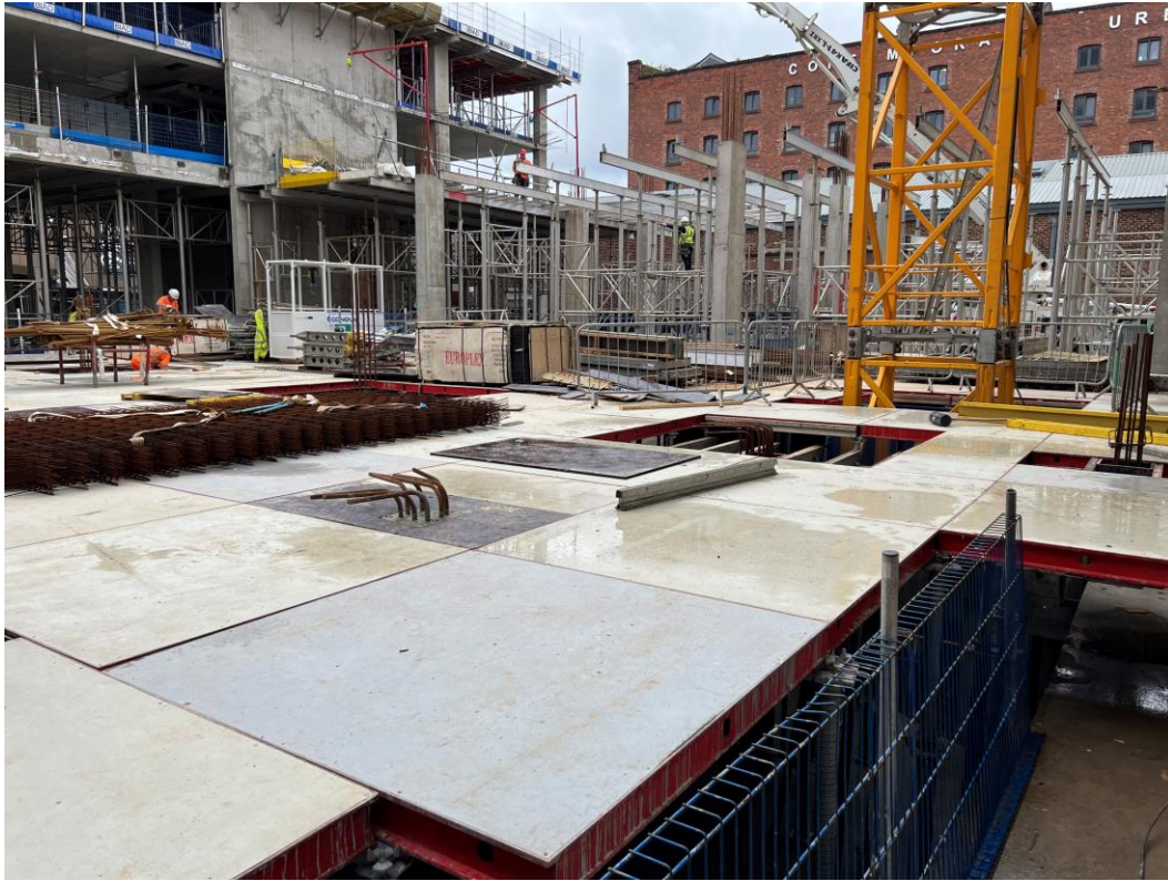
Zone C – Shuttering in place for Ground Floor slab pour
