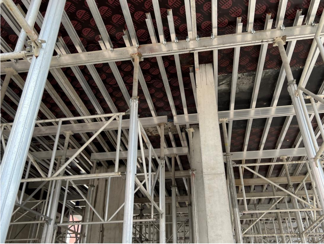
Formwork for slab casting in place
