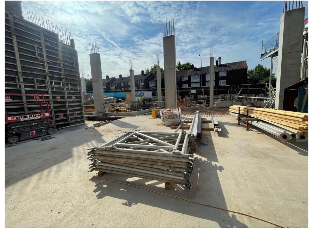
Ground Floor columns cast
