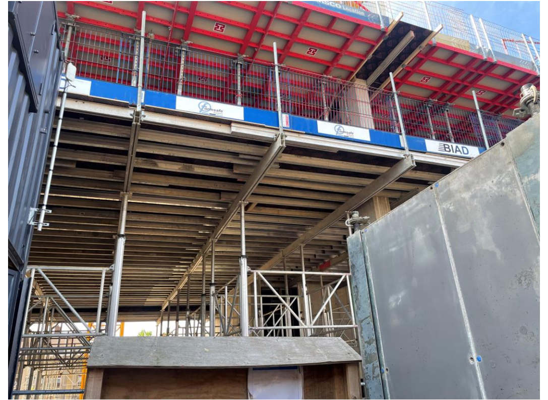
Formwork for upper floor slabs installed
