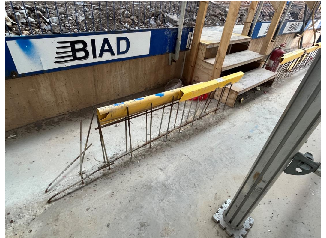
Reinforcement for concrete upstand
