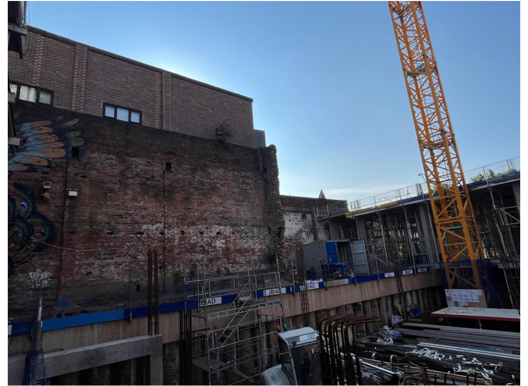
Contiguous wall installed
