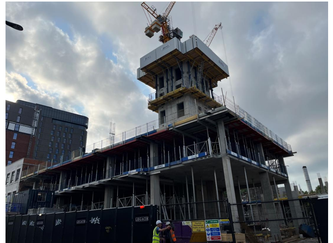
Zone A – reinforced concrete frame construction ongoing
