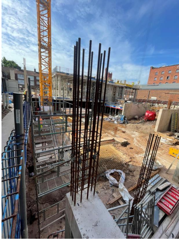
Reinforcement for columns
