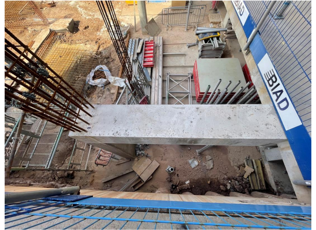
First Floor beam cast
