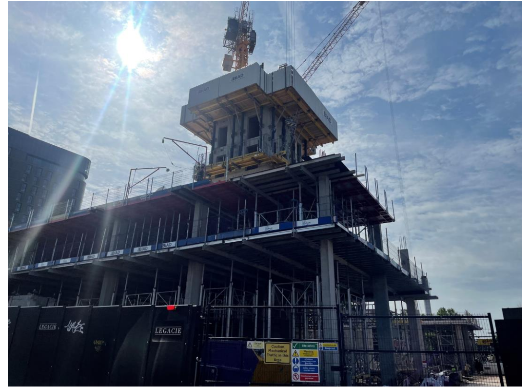
Zone A – reinforced concrete frame construction ongoing
