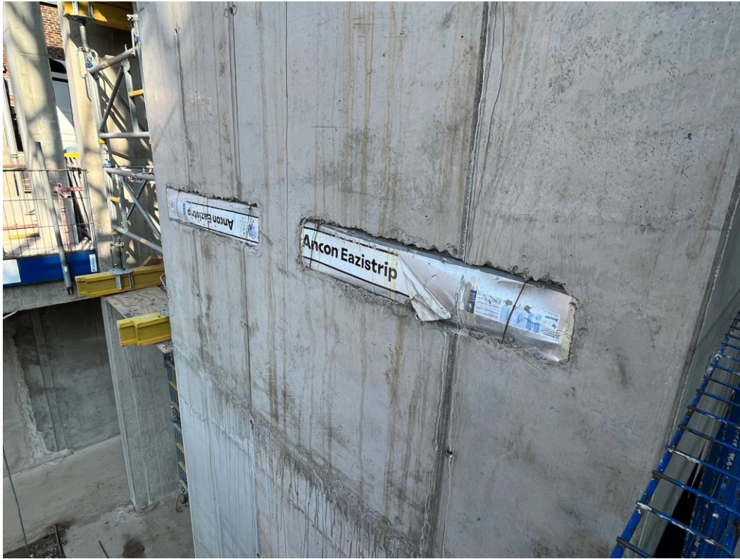
Reinforcement continuity installed
