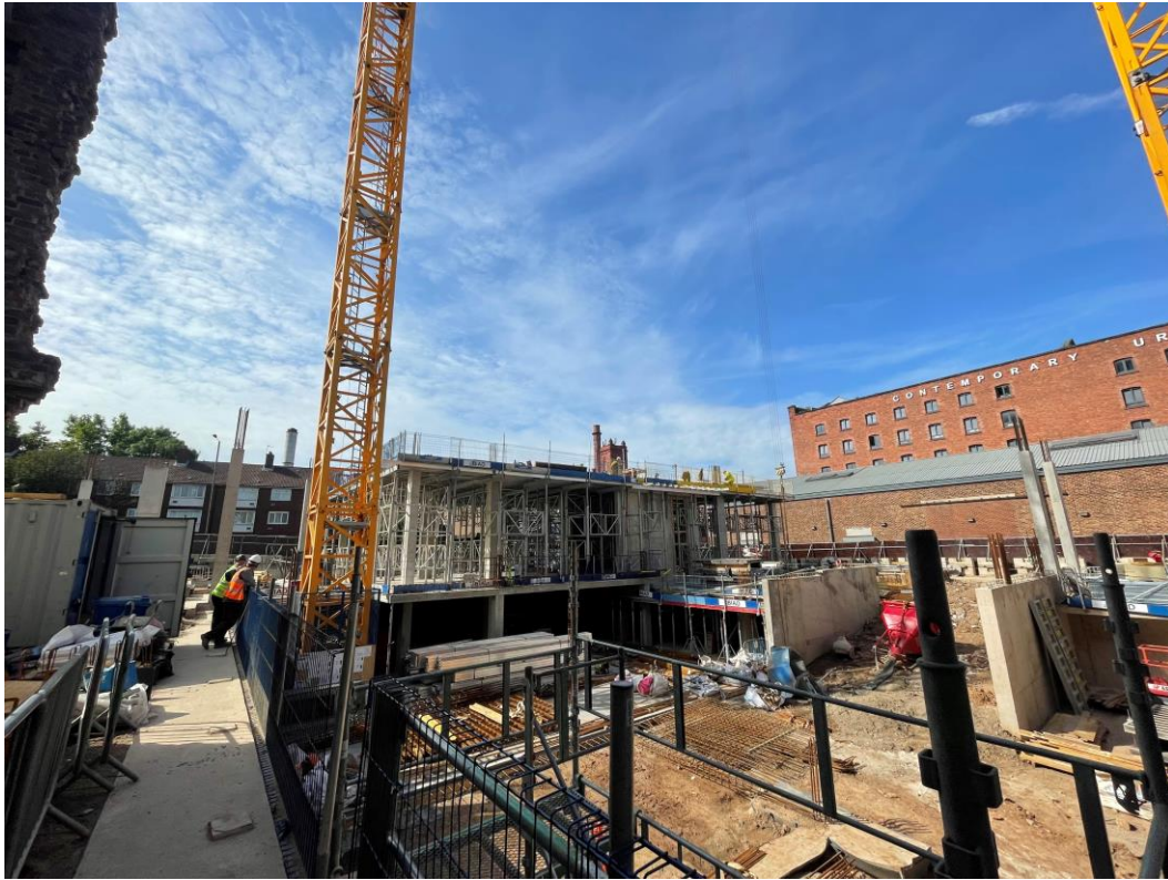
Zone C – Reinforced frame construction ongoing
