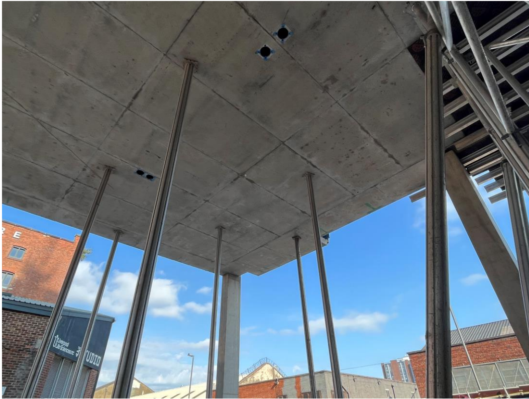
Formwork removed to first floor slab
