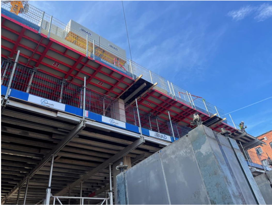
Formwork for upper floor slabs installed
