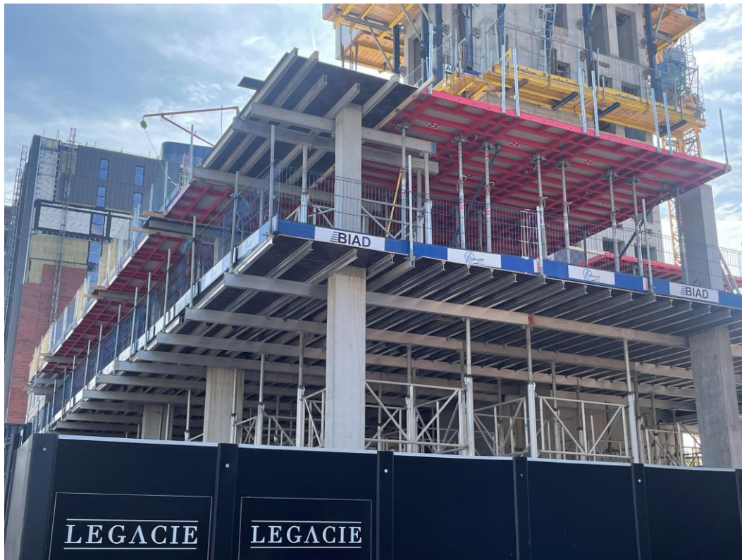
Zone A – reinforced concrete frame construction ongoing
