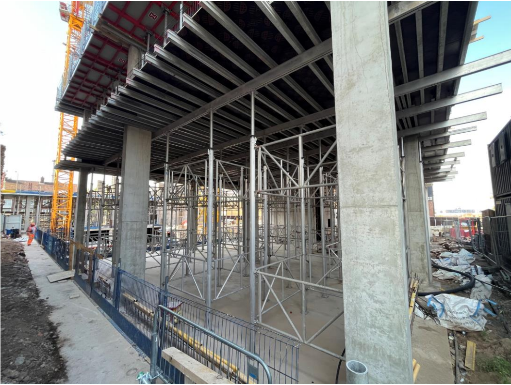
Ground floor columns cast
