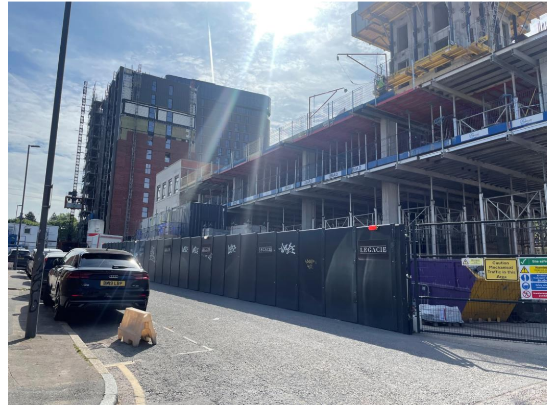
New site hoarding installed
