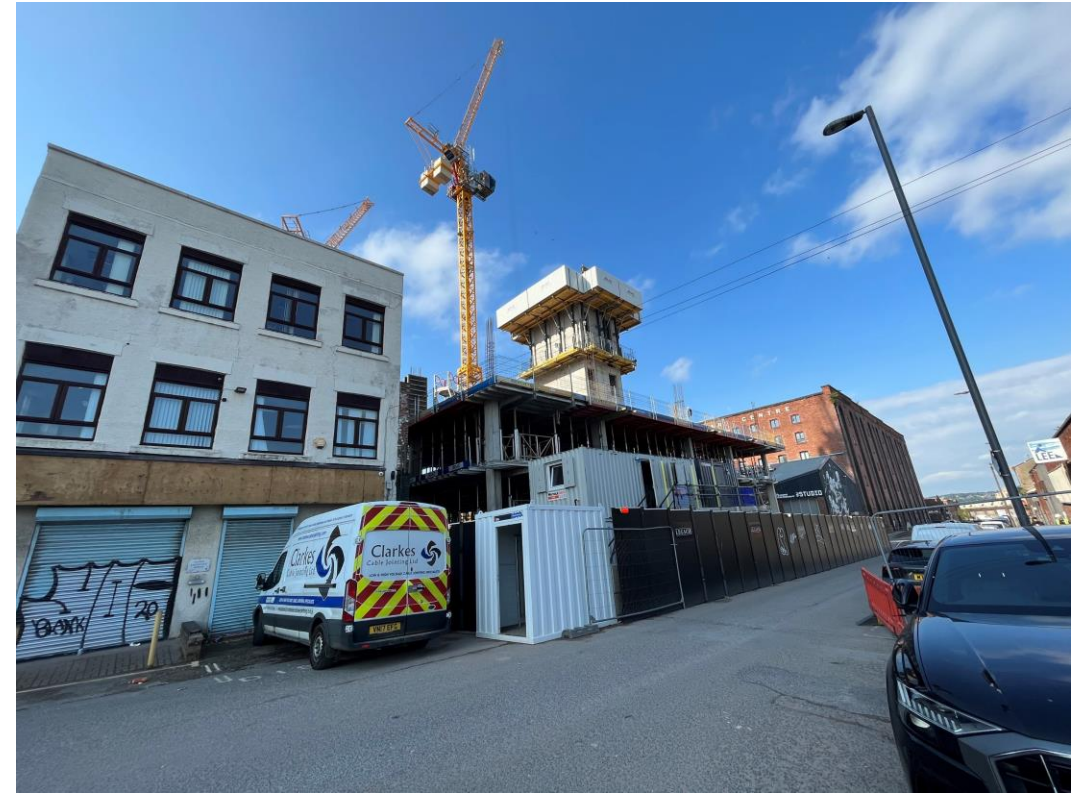
Zone A – reinforced concrete frame construction ongoing
