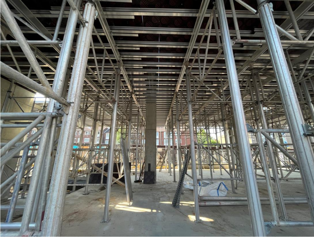
Formwork for floor slab casting in place
