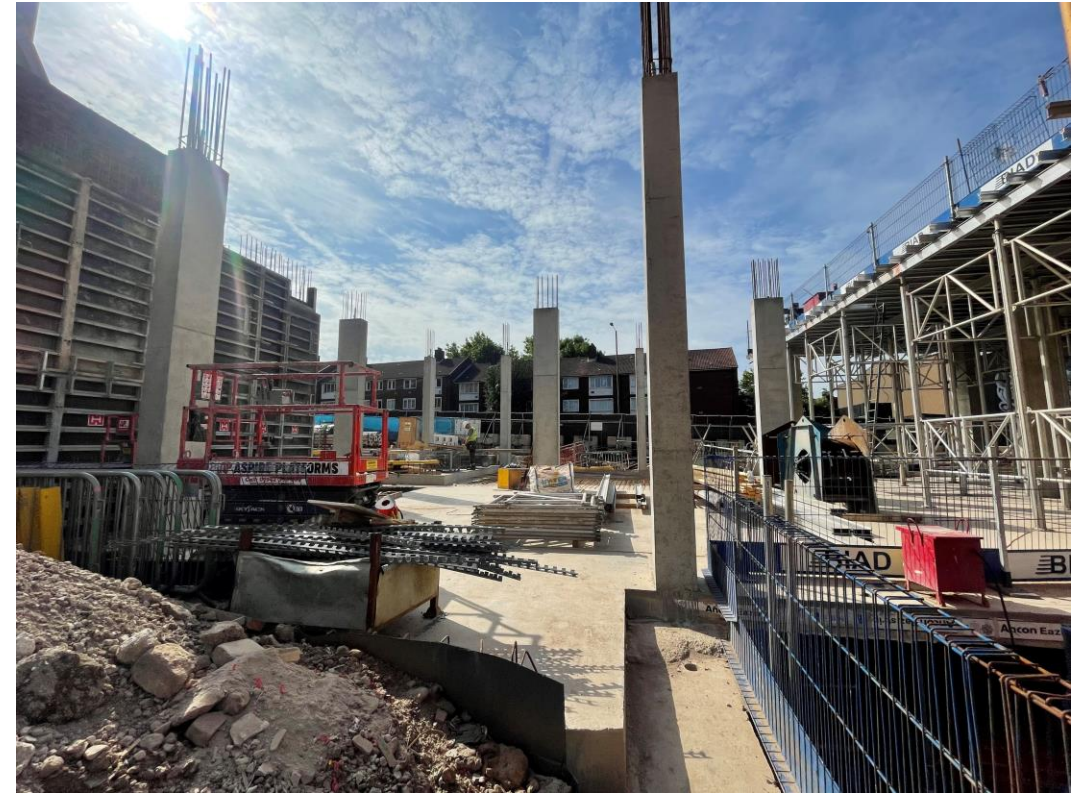
Ground floor column
