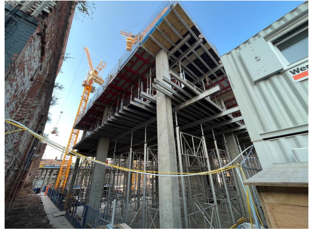
Zone A – reinforced concrete frame construction ongoing
