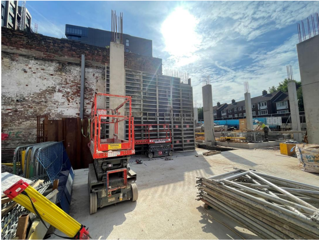
Formwork for retaining wall installed
