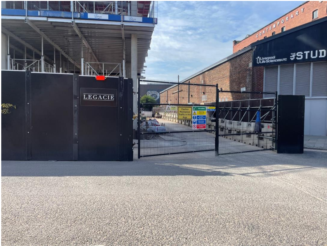
Site access gate from Greenland Street
