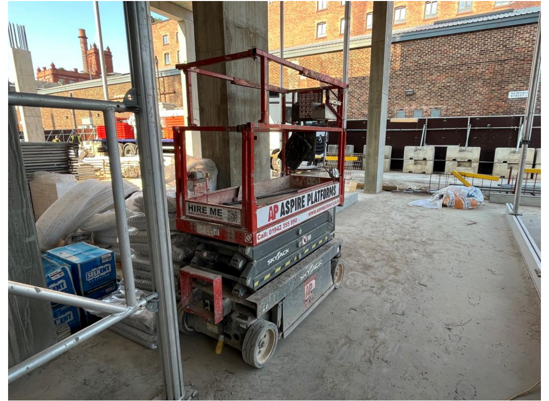
Scissor lift on site
