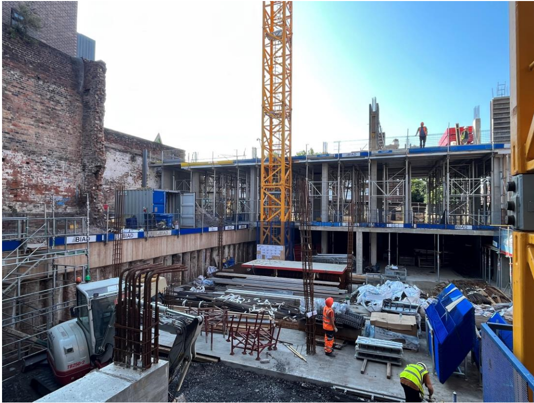
Zone C – Reinforced frame construction ongoing
