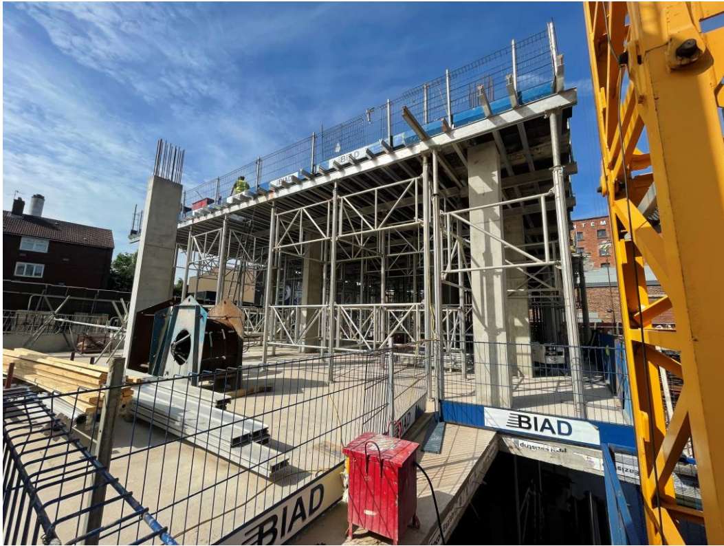
Zone C – Reinforced frame construction ongoing
