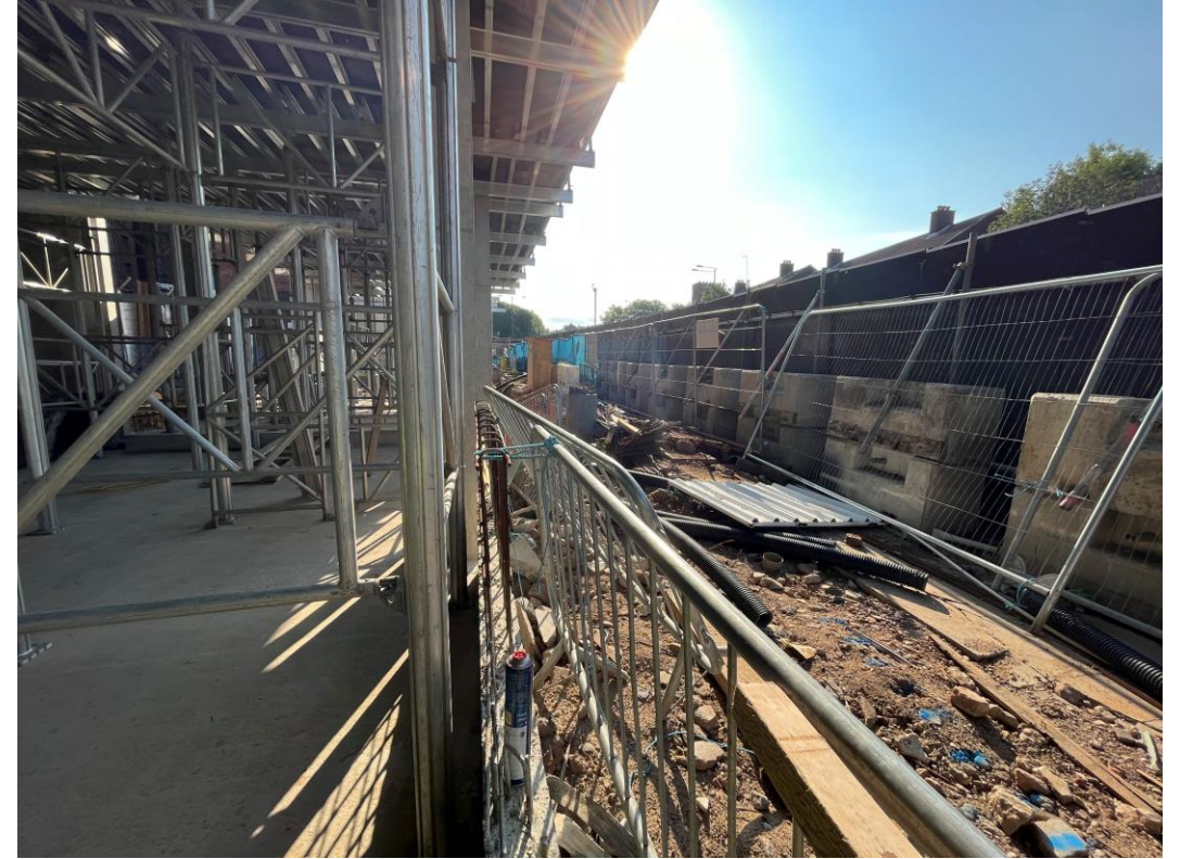
Formwork for floor slab casting in place
