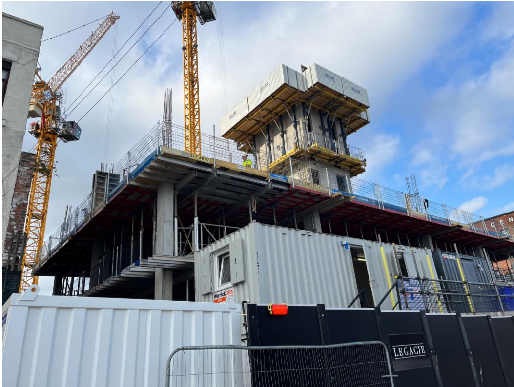
Zone A – reinforced concrete frame construction ongoing
