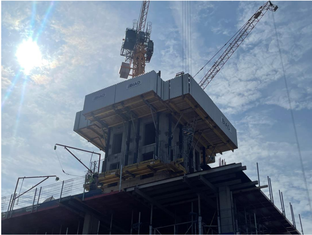
Staircore 2 under construction
