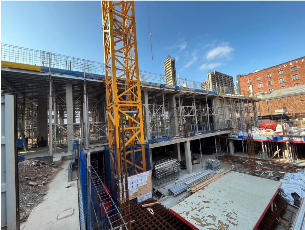
Zone C – Reinforced frame construction ongoing
