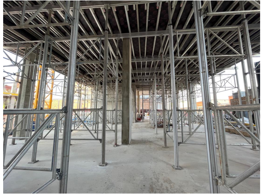
Formwork for floor slab casting in place
