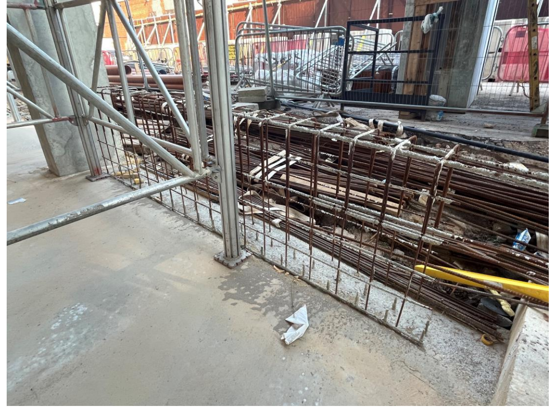
Reinforcement for concrete upstand
