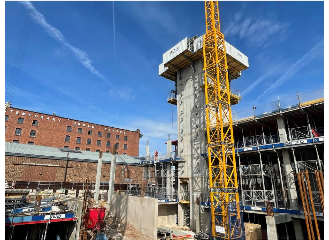
Zone A – Reinforced frame construction ongoing
