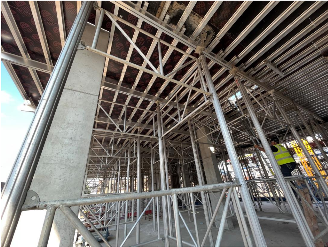
Formwork for floor slab casting in place
