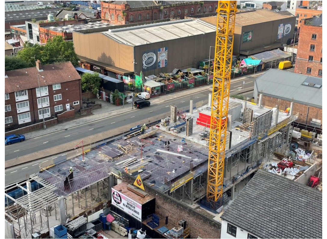
Reinforcement installation to first floor slab
