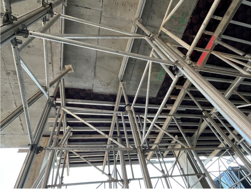
Formwork for floor slab casting in place
