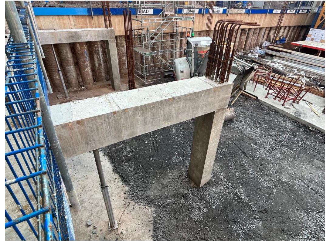
Reinforce concrete beam and column cast
