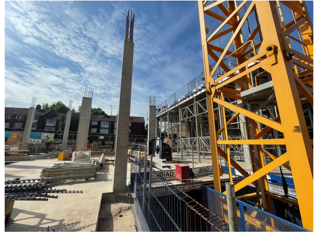
Ground floor columns cast
