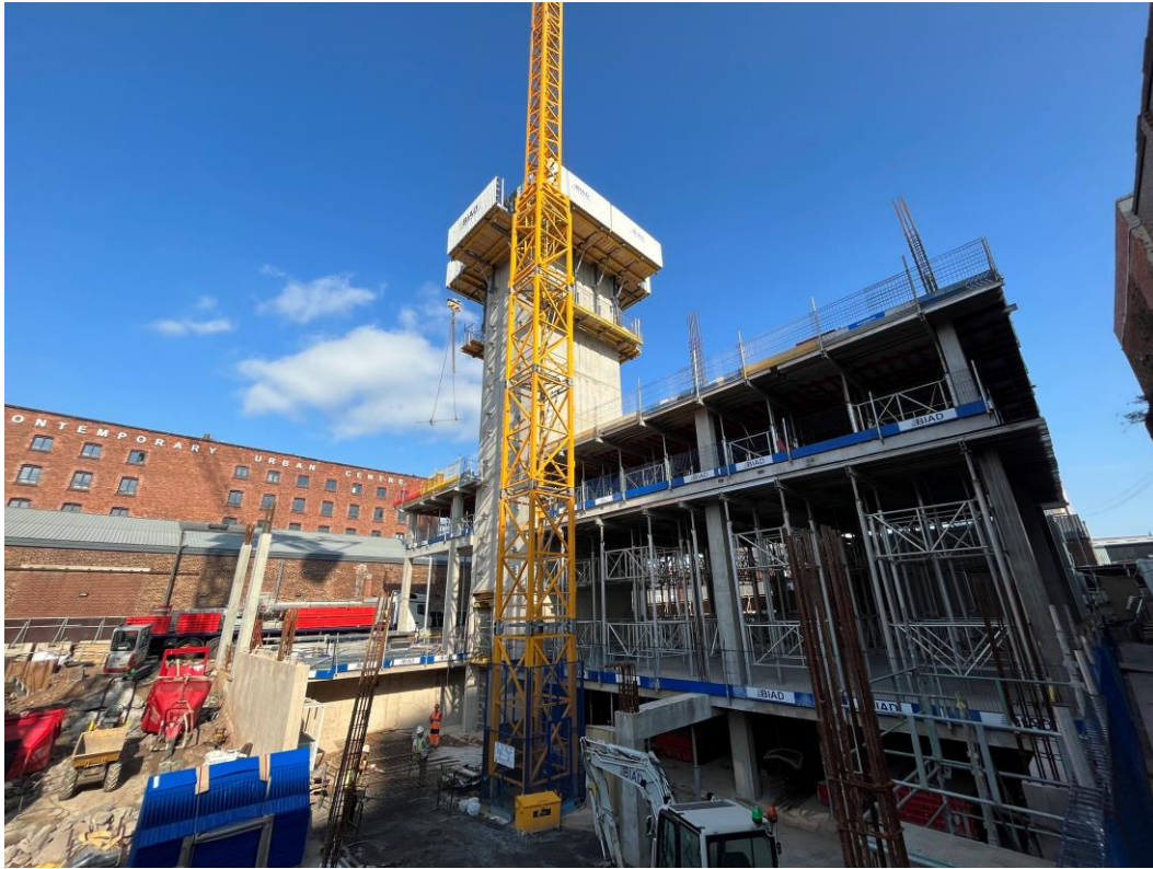
Zone A – Reinforced concrete frame construction ongoing
