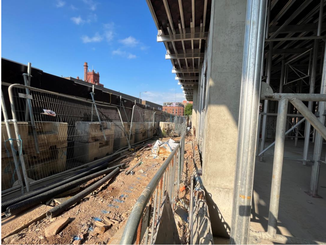
Formwork for floor slab casting in place
