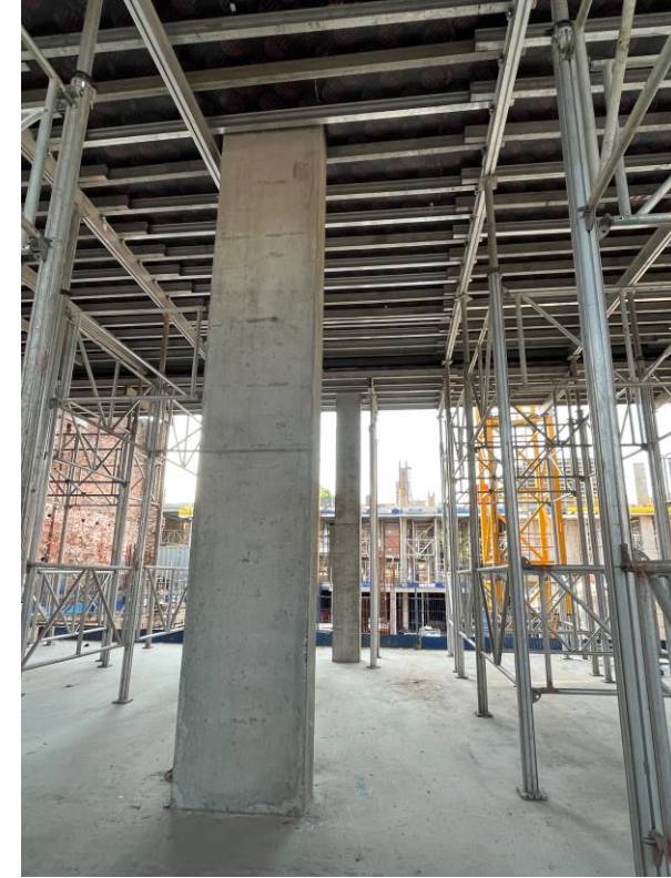
Ground floor columns cast
