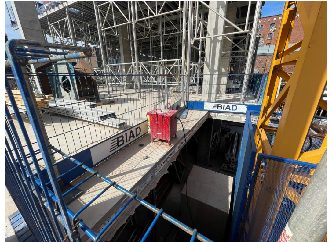
Ground floor slab cast
