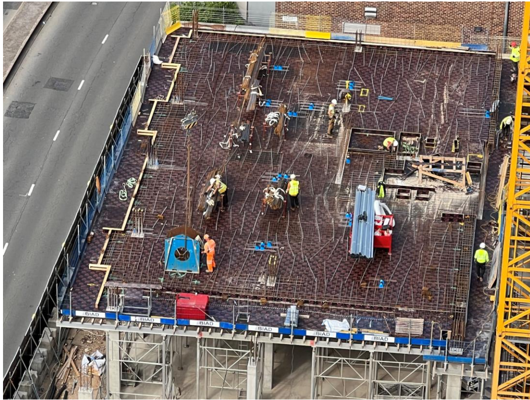
Reinforcement installation to first floor slab
