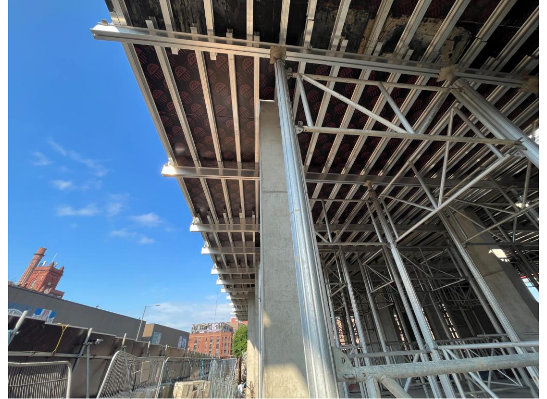
Formwork for floor slab casting in place
