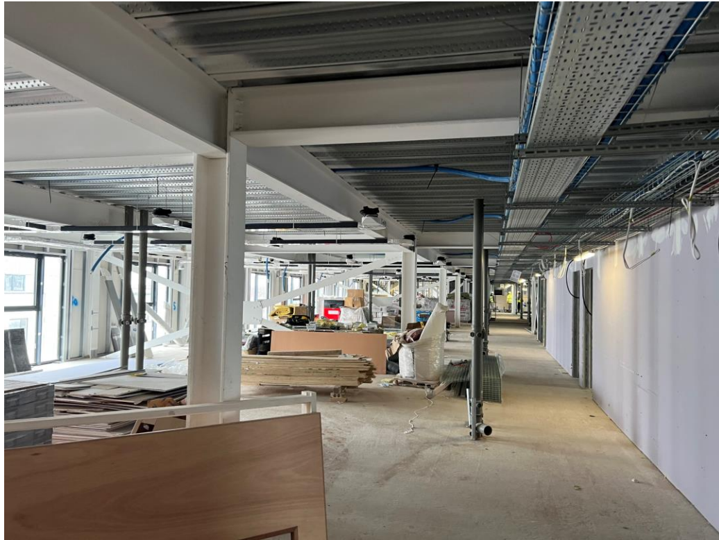
Residential Block – General site activity
