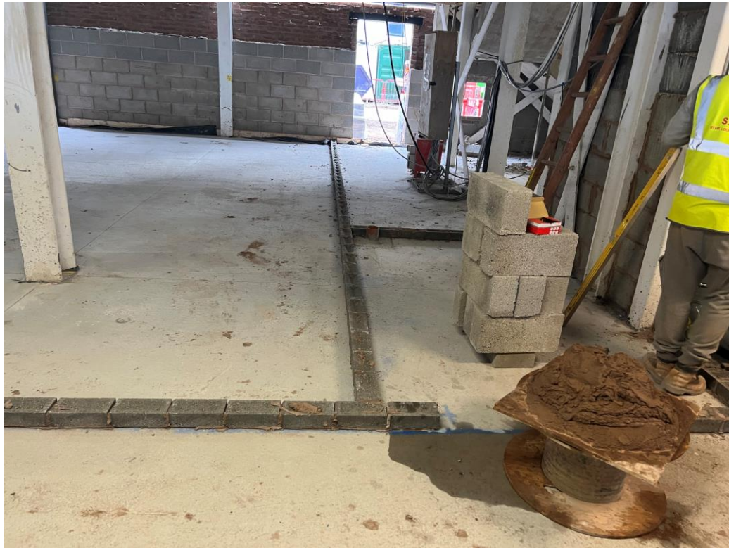
Internal blockwork walls
