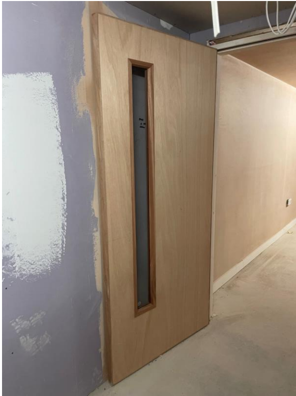
Student Wing – Internal fire doors installation
