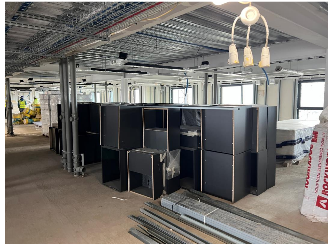
Kitchen units loaded for installation
