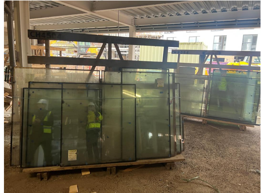
Material storage – Glazing units
