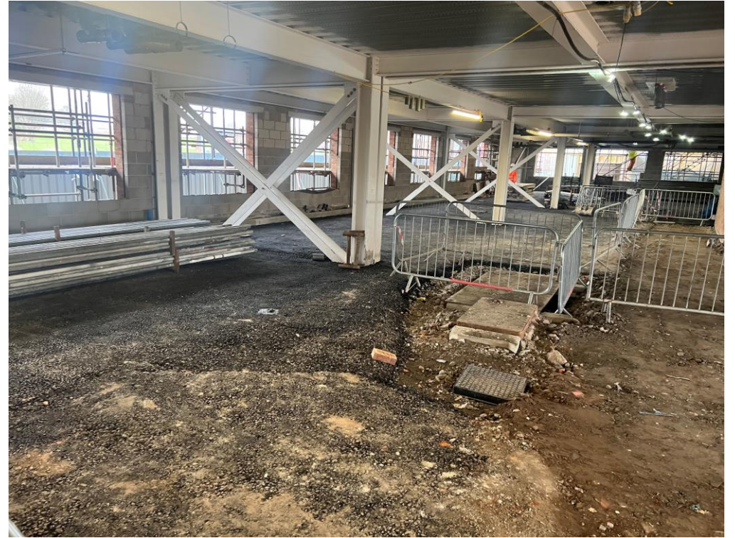
Installation of tarmac road surface commenced
