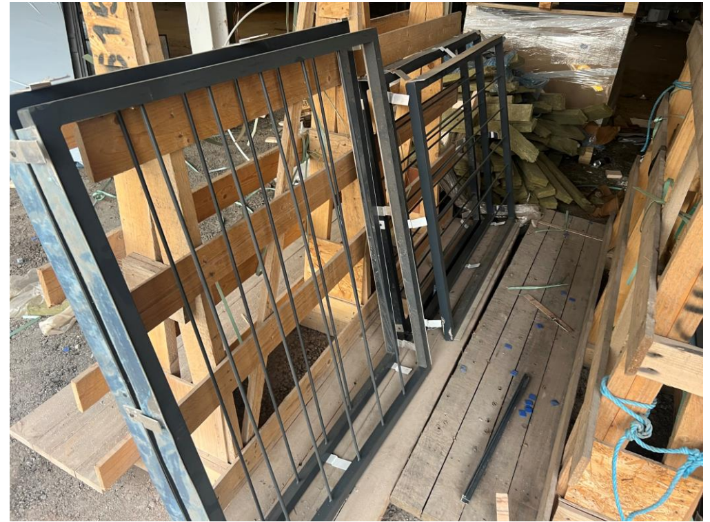
Vent grills for undercroft parking area
