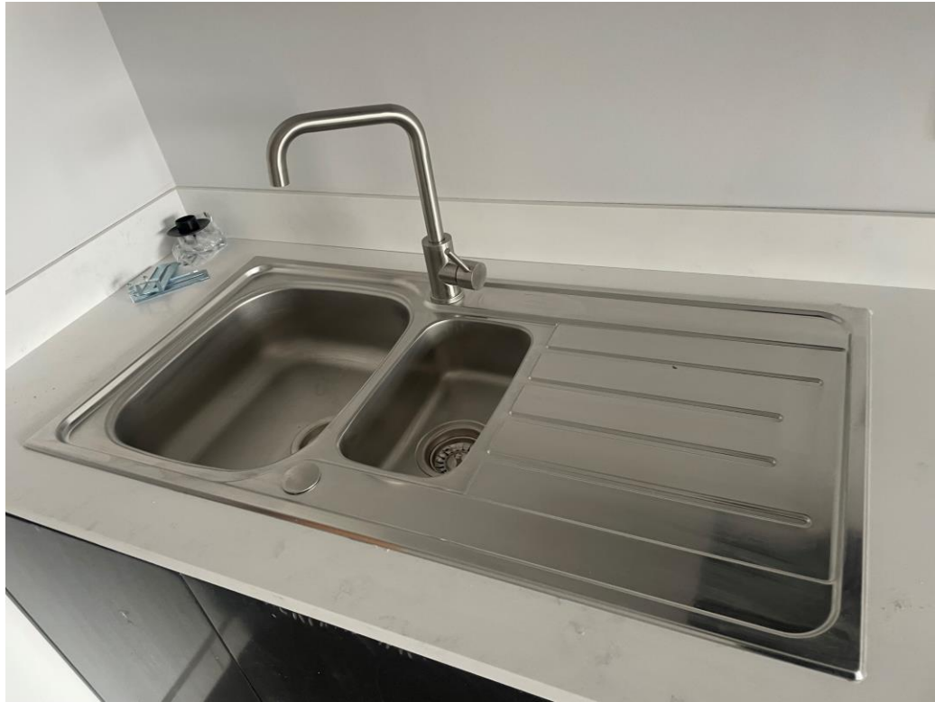
Student Wing – Kitchen sink and tap installation
