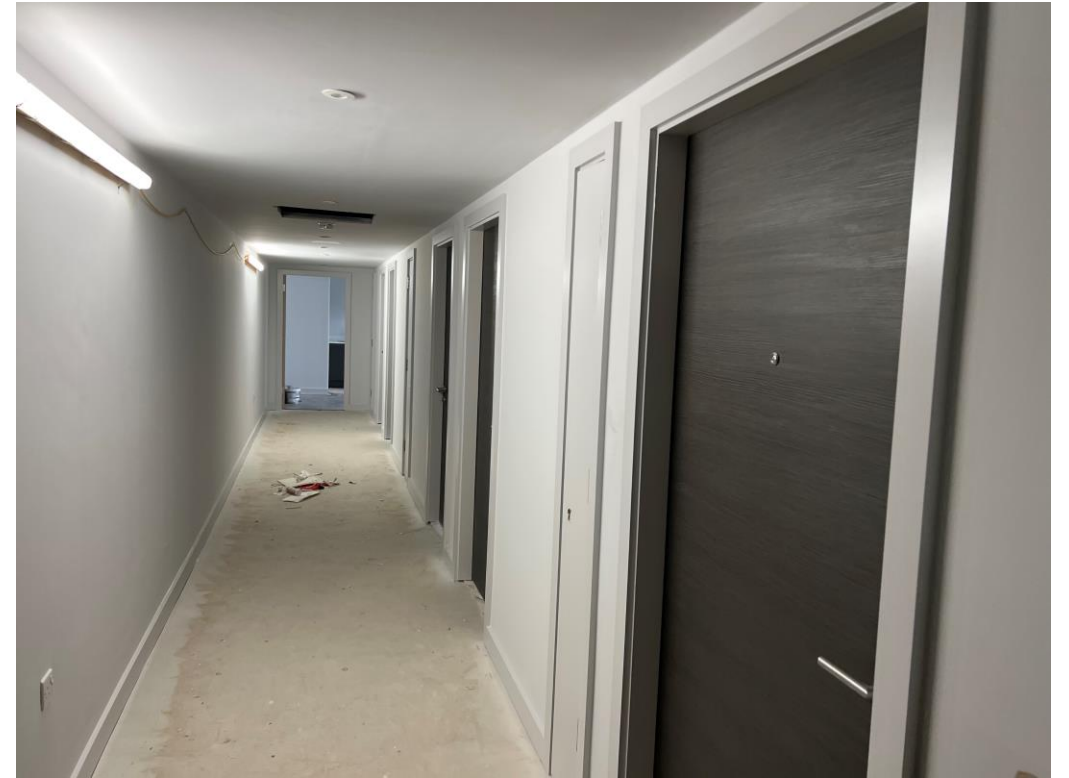
Student Wing – Internal finishes on-going
