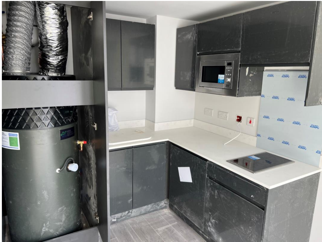
Student Wing – Kitchen installed
