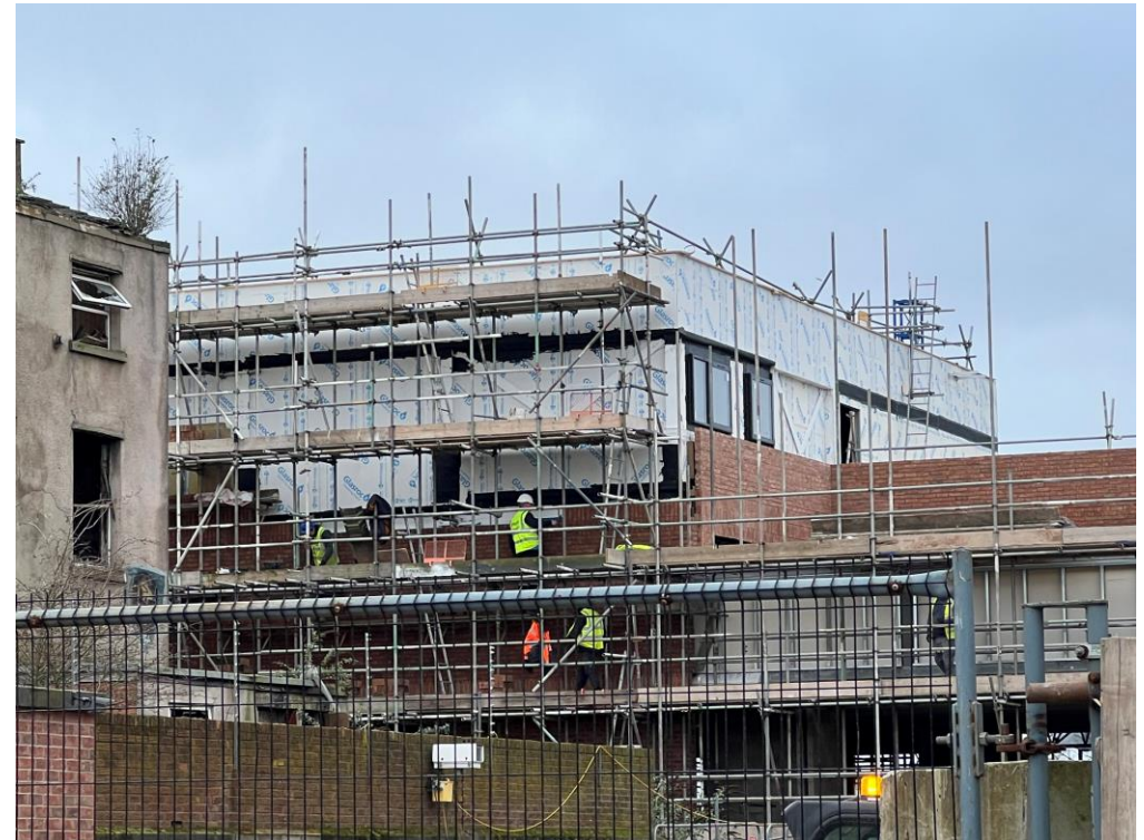
Commercial Block – Brickwork Installation
