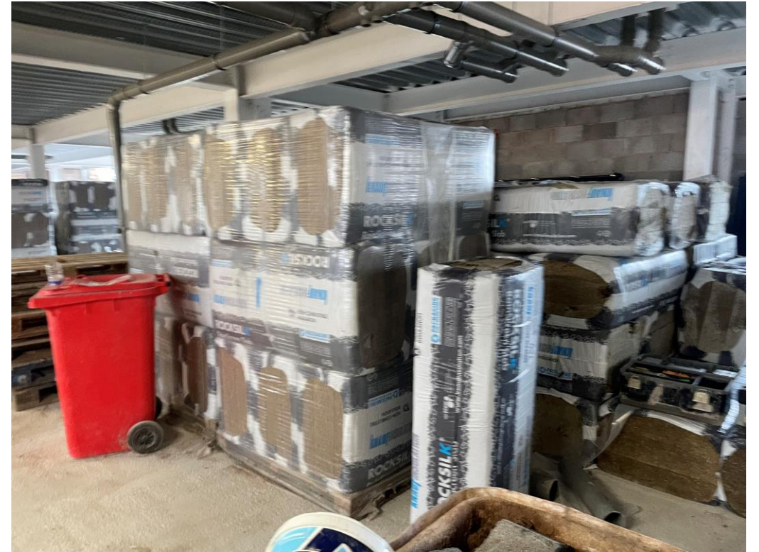
Material storage – Insulation
