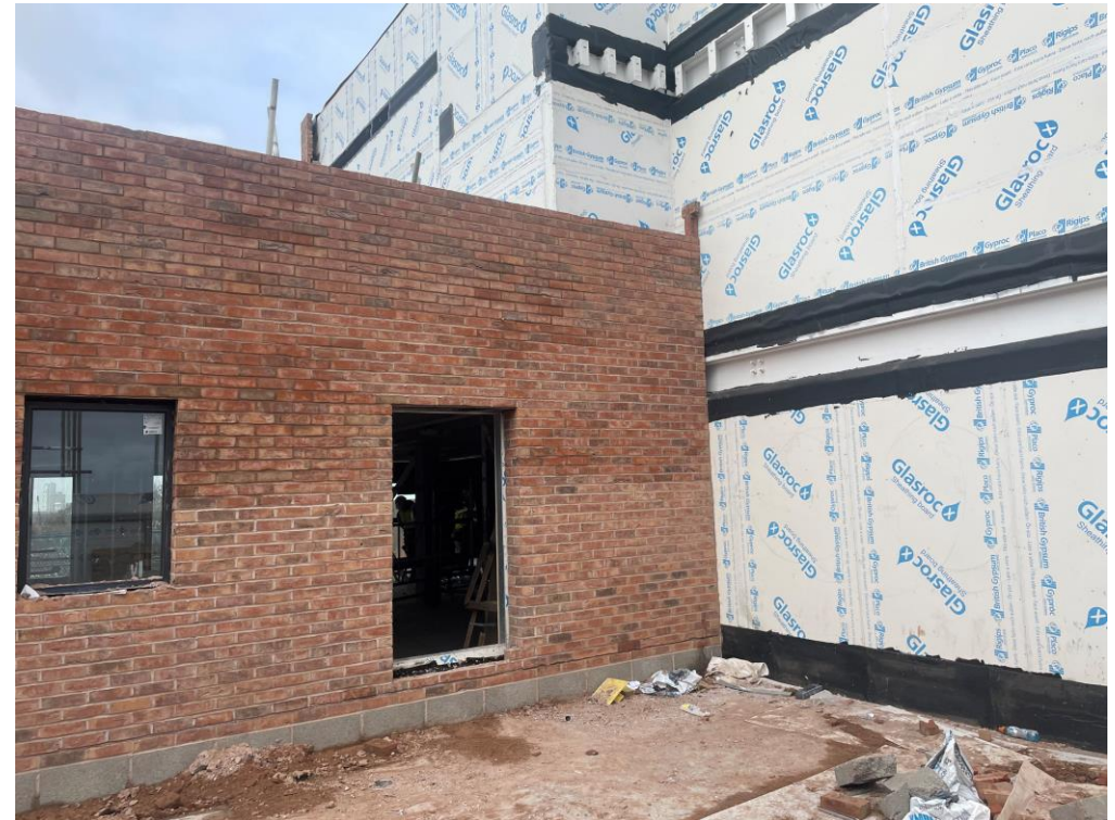
Brickwork installation ongoing
