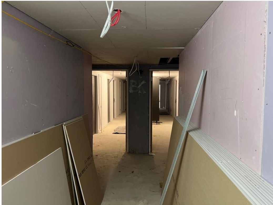
Student Wing – Internal finishes on-going
