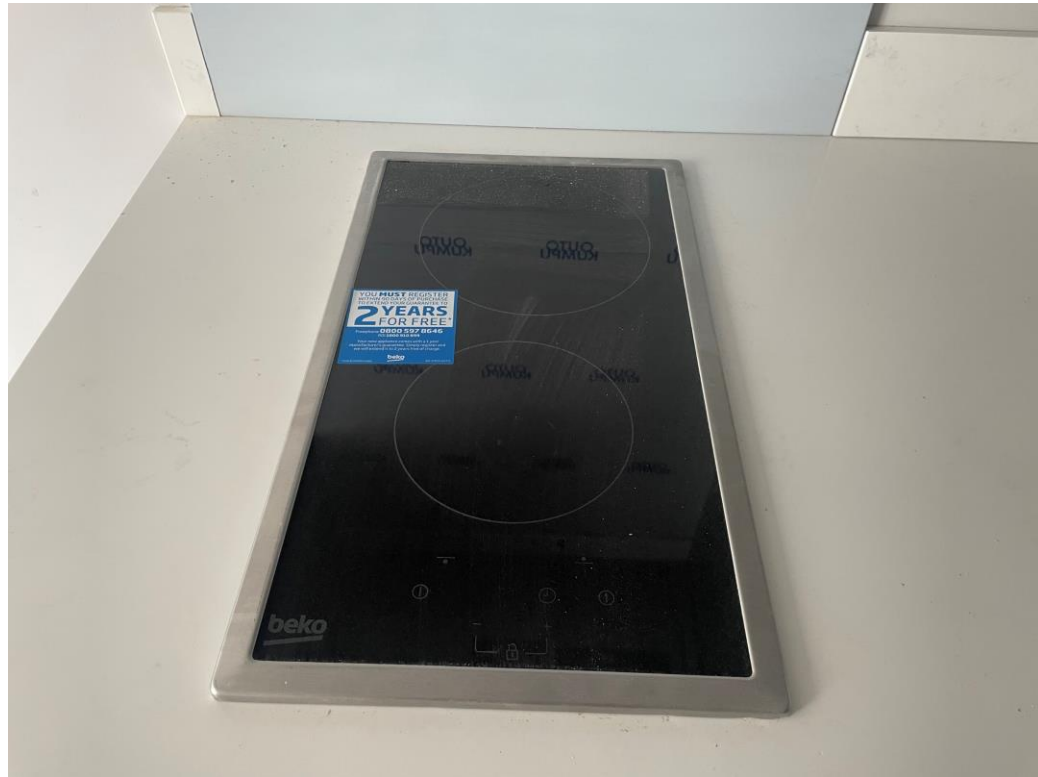
Student Wing – Kitchen appliance installation
