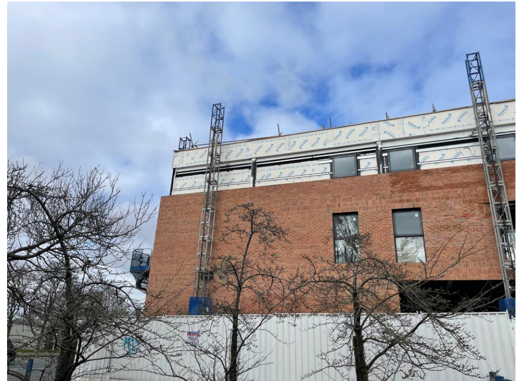
Brickwork installation ongoing
