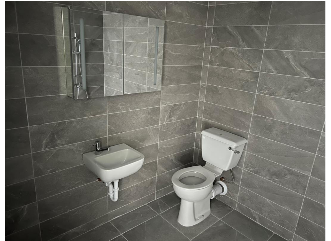
Student Wing – Sanitaryware installation
