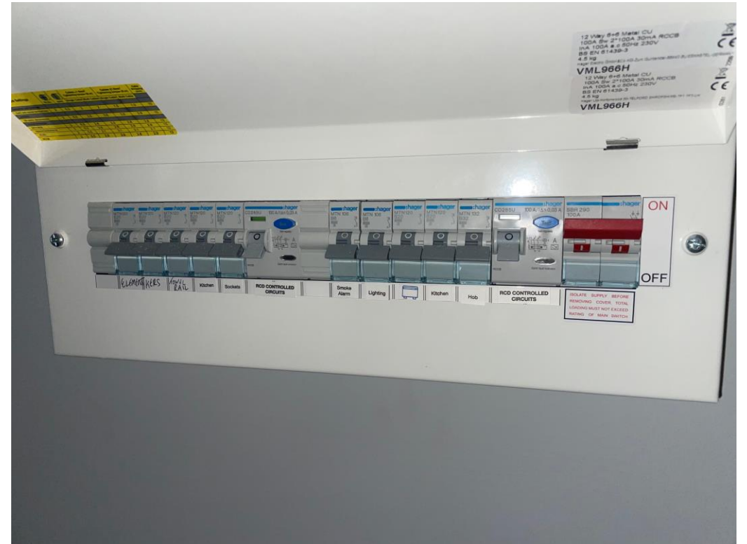
Student Wing – Distribution board installation
