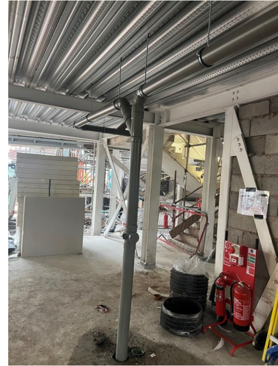
Internal drainage installation on-going
