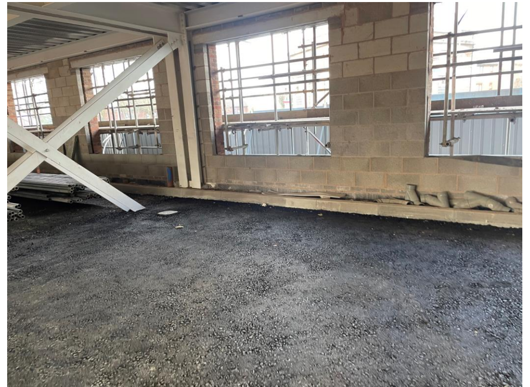
Tarmac laid to undercroft parking spaces
