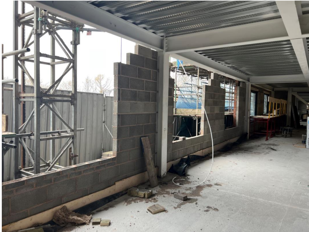
Installation of blockwork walls on-going
