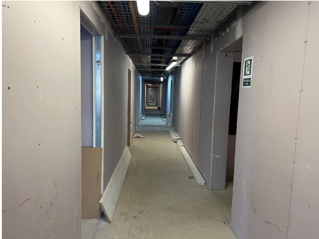
Residential Block – Internal finishes on-going
