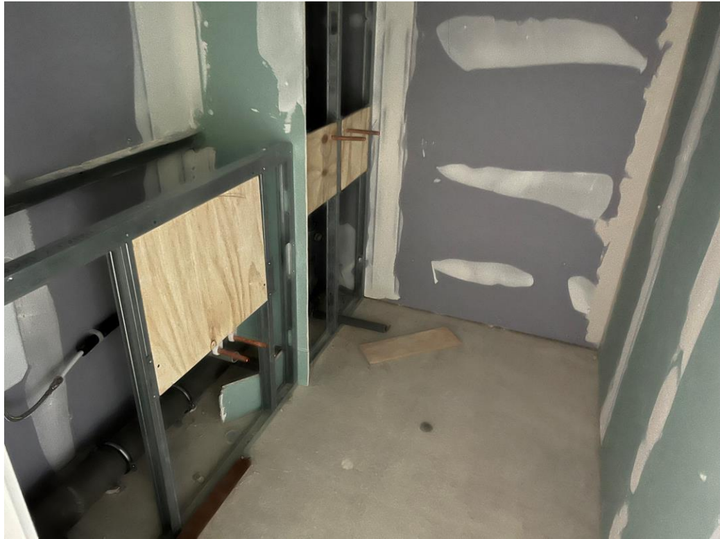
Residential Block - IPS Installation on-going
