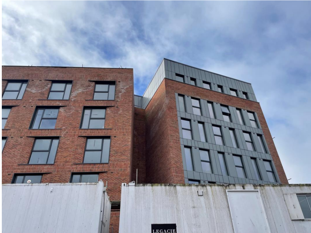
Rainscreen cladding installation complete
