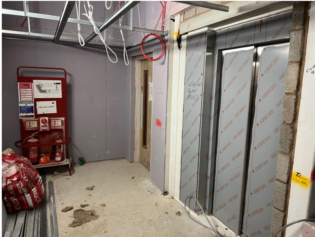
Lift installation on-going
