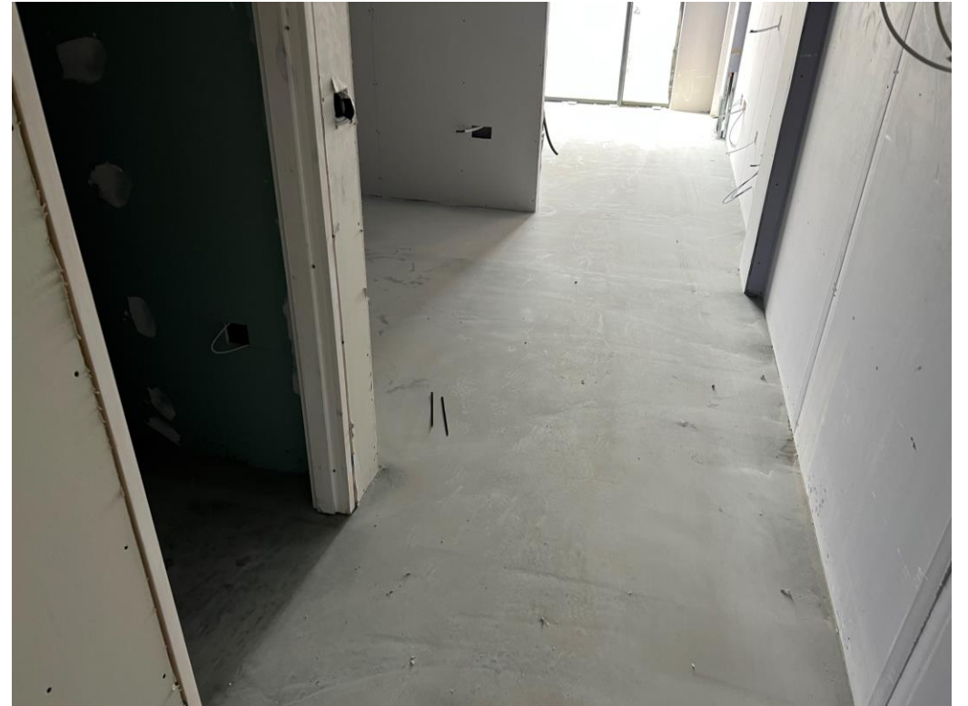
Residential Block - Latex screed applied to floors
