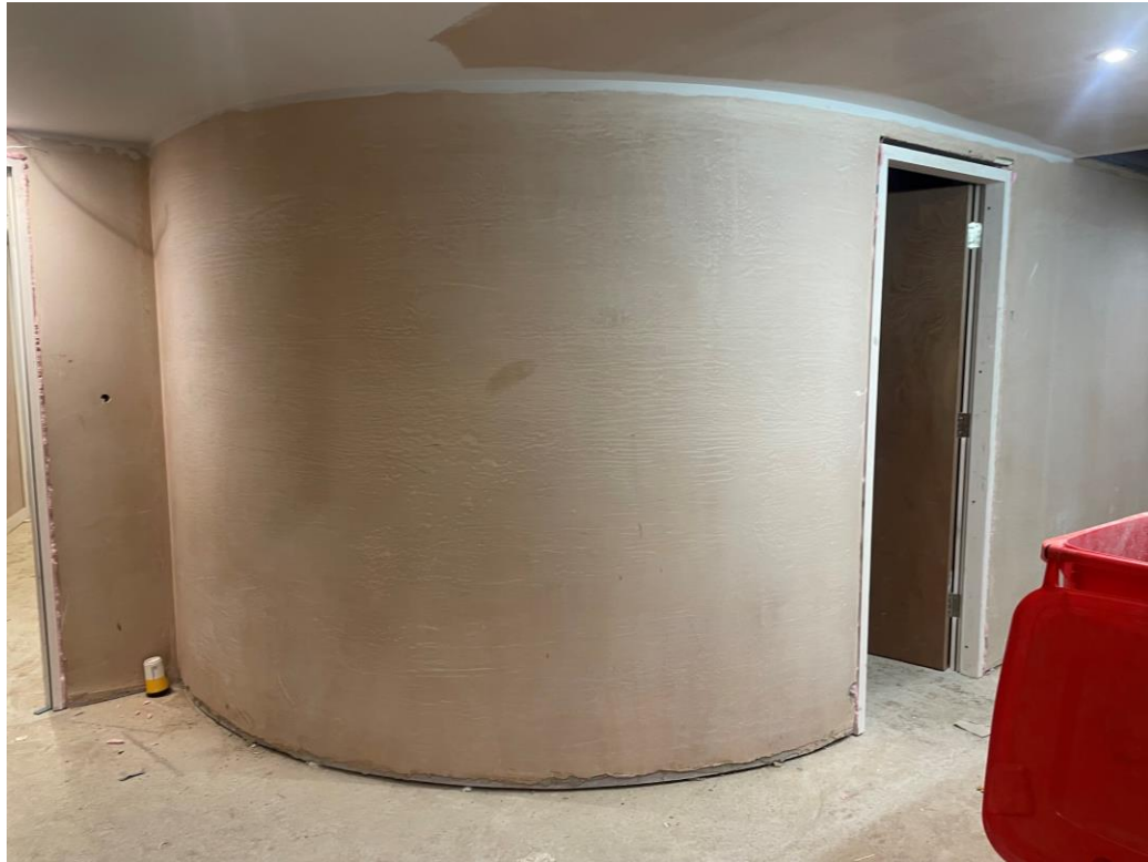
Residential Block – Internal finishes on-going
