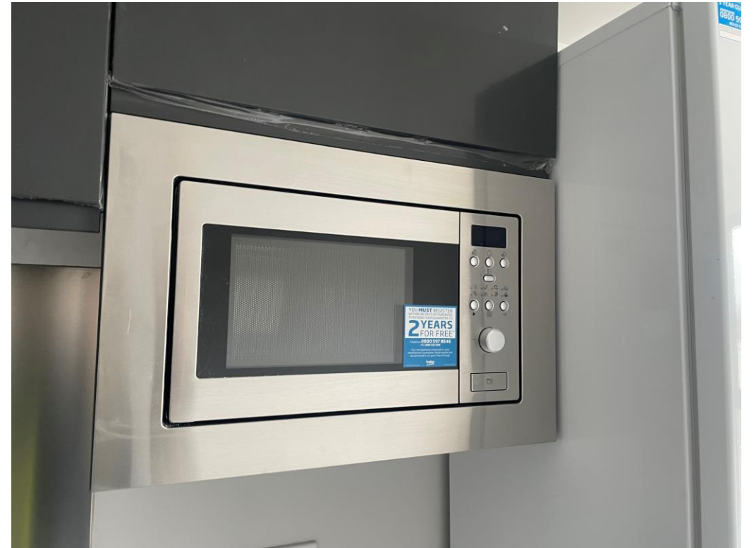
Student Wing – Kitchen appliance installation
