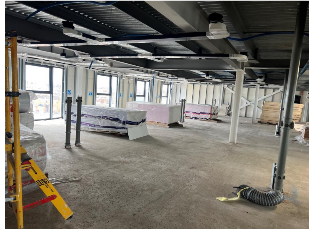
Residential Block – General site activity
