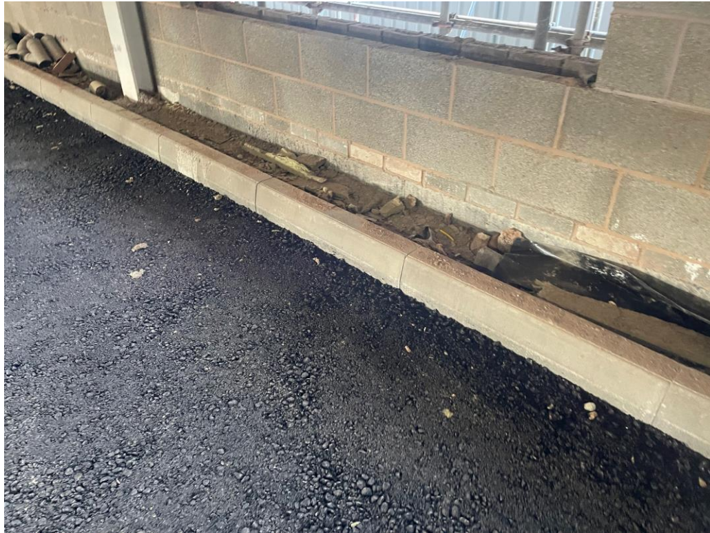
Kerbing installation commenced
