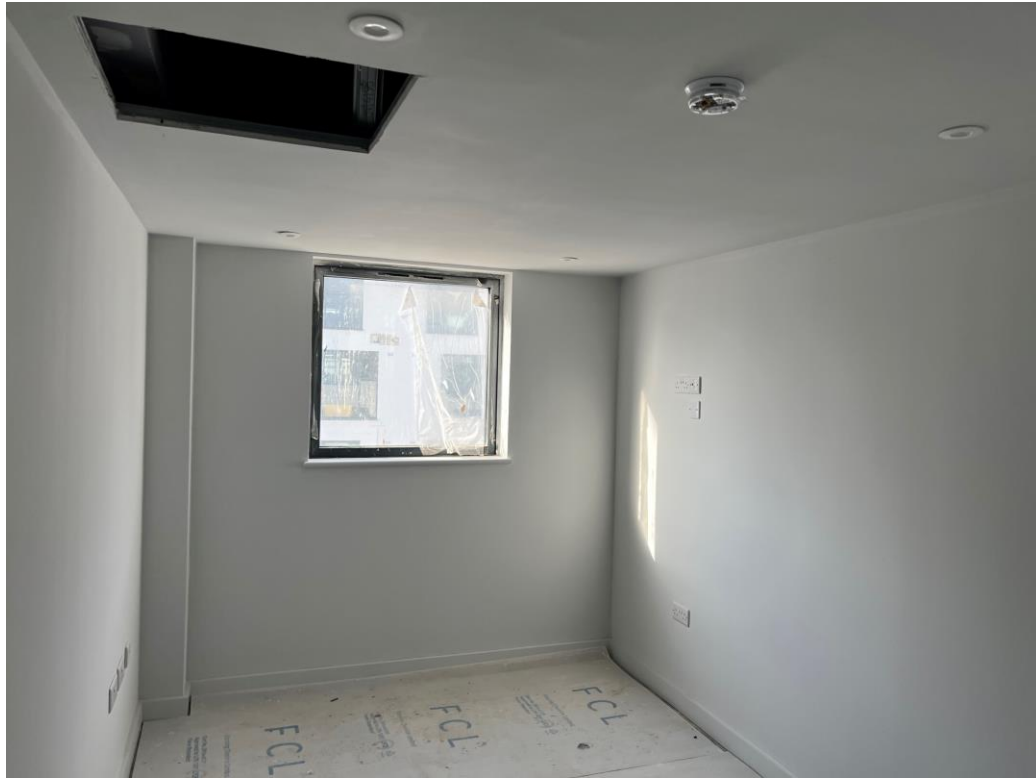
Student Wing – Internal finishes complete
