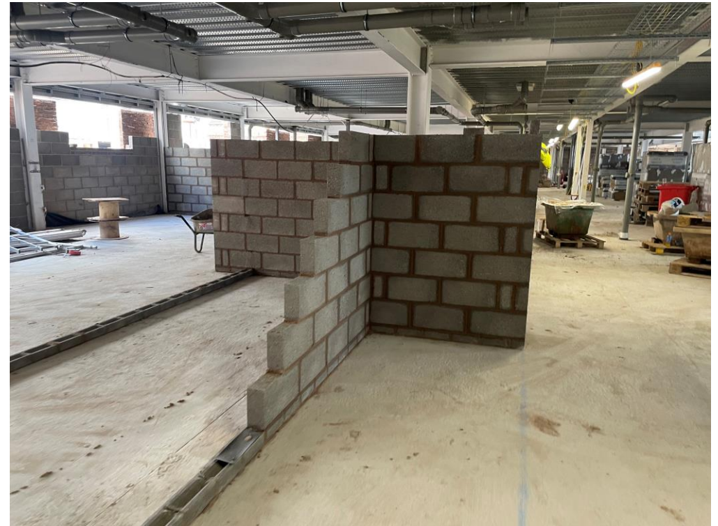
Ground Floor blockwork ongoing
