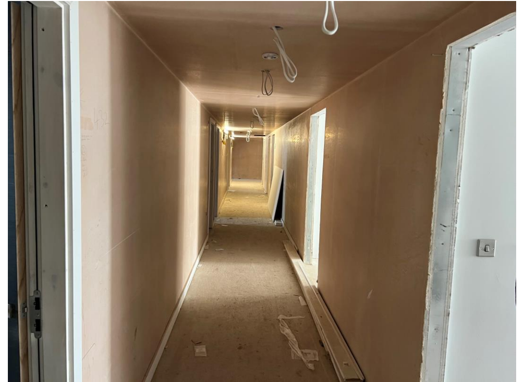
Student Wing – Internal finishes on-going
