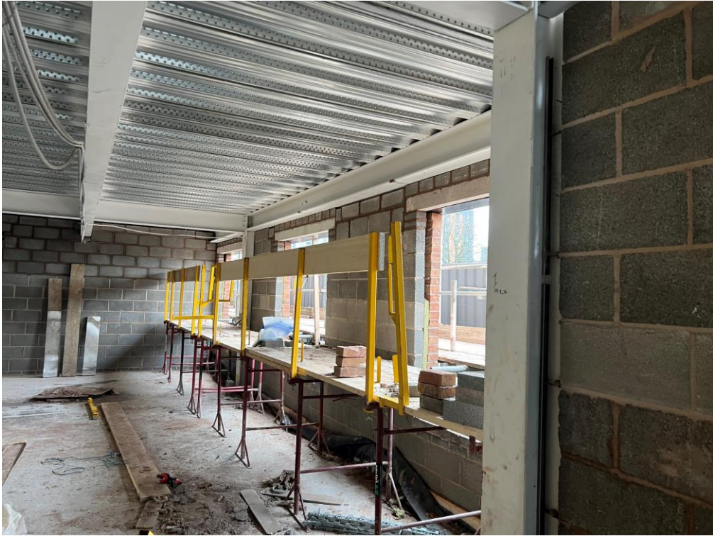
Installation of blockwork walls on-going
