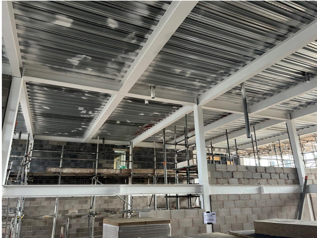
Installation of blockwork walls on-going
