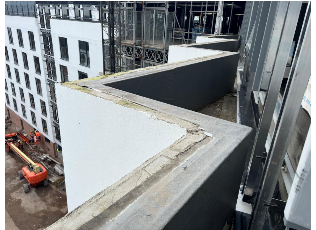
Parapet wall awaiting capping's
