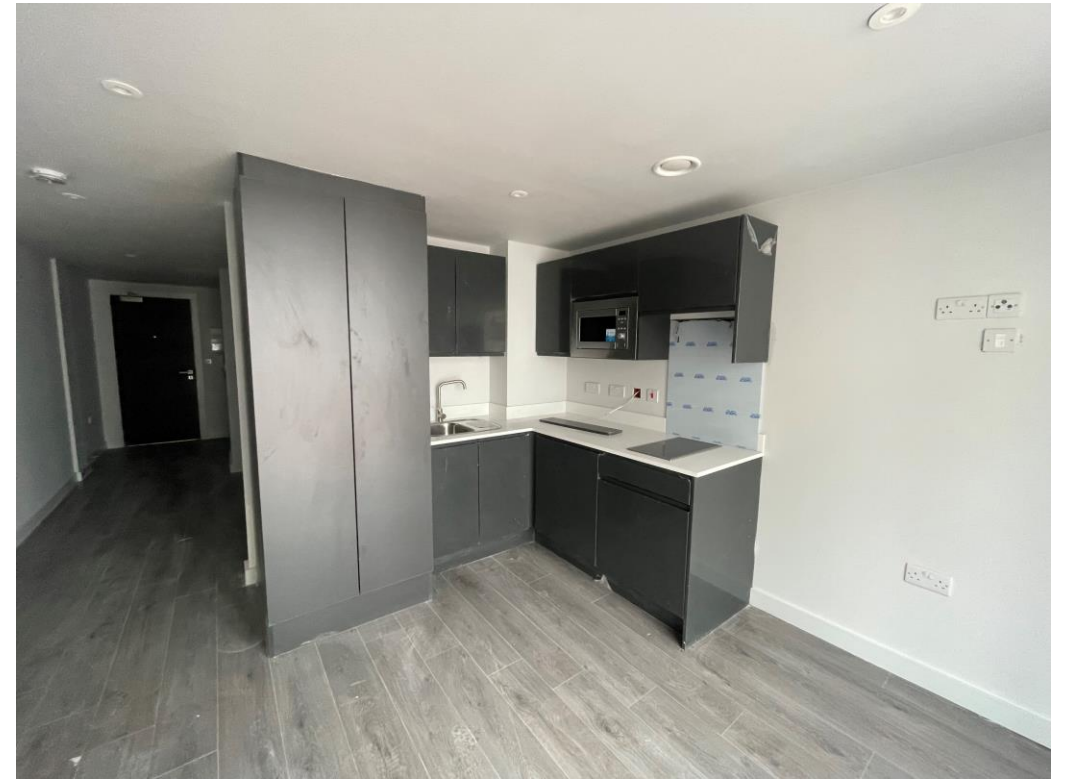
Student Wing – Kitchen installation
