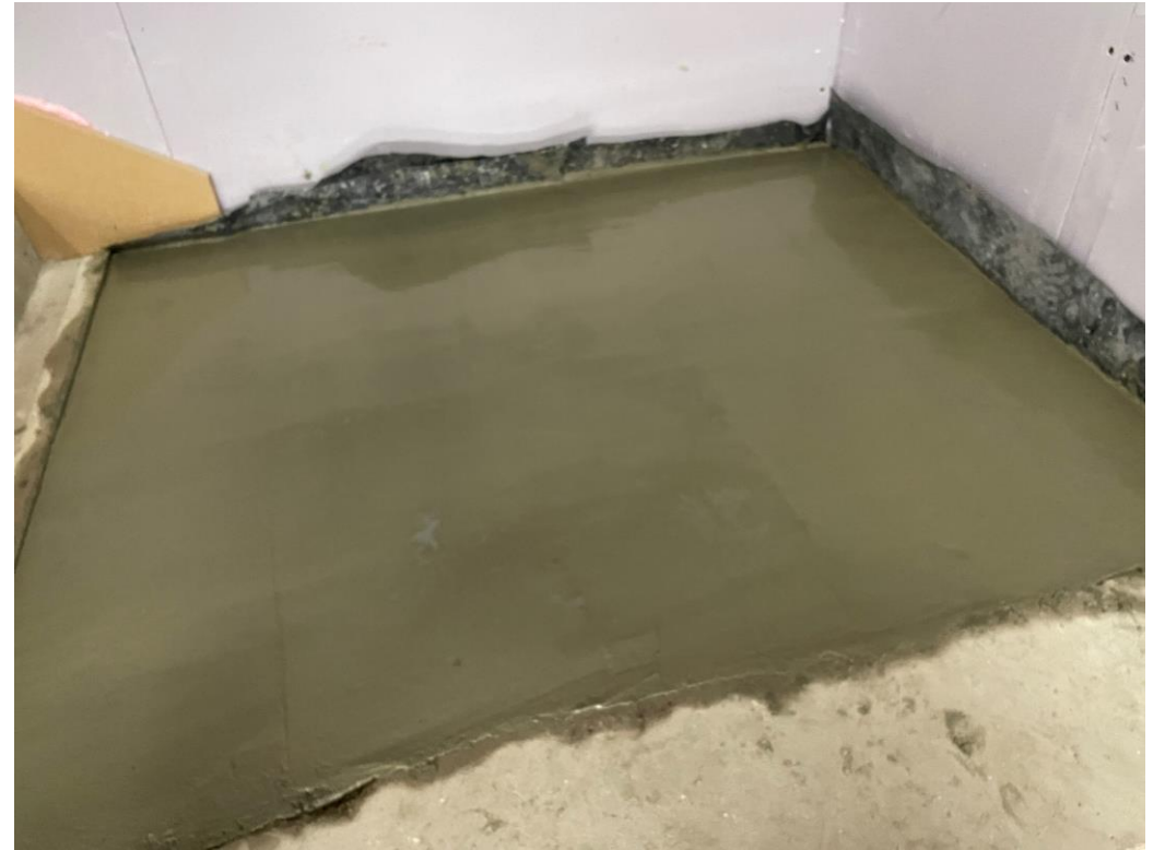
Residential Block – Concrete slab levelling to staircase landing
