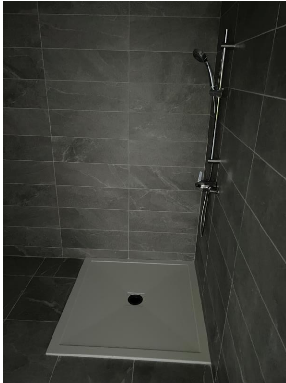
Student Wing – Shower tray installation
