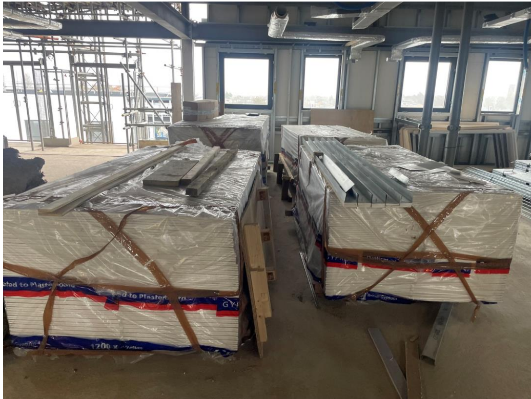
Material storage – Plaster Boarding
