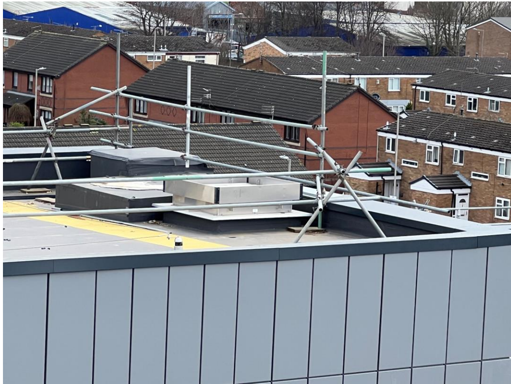
Capping installed
