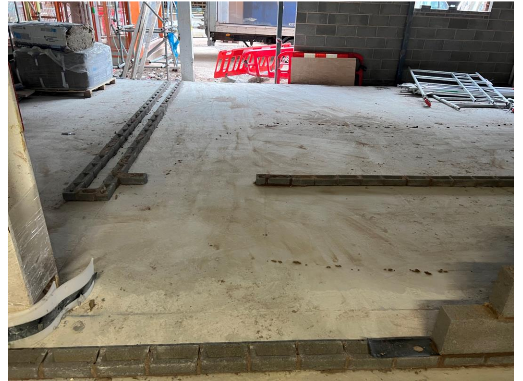
Internal blockwork walls
