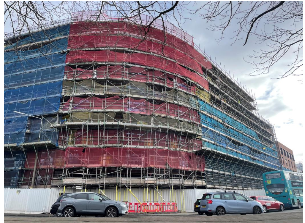
Brunswick Road – Site View
