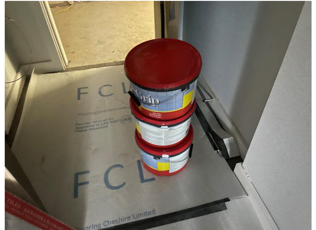
Material storage – Tile adhesive
