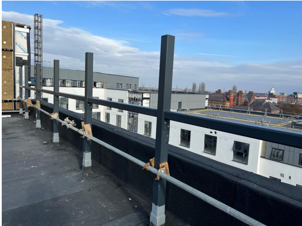
Balustrade installation ongoing
