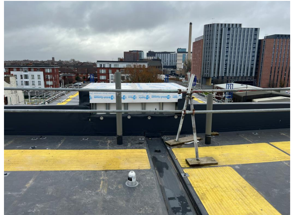
Balustrade installation ongoing
