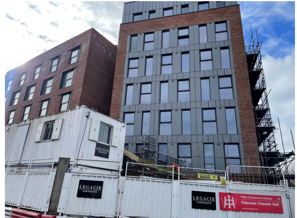
Walker Street - Site view
