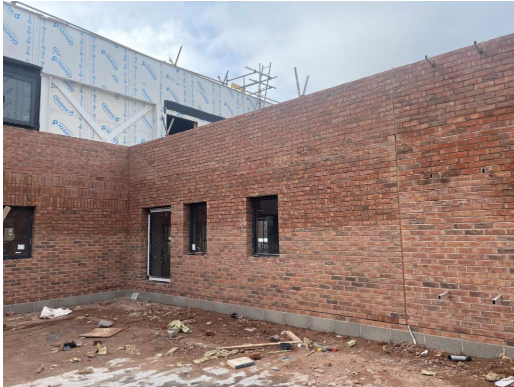
Brickwork installation ongoing
