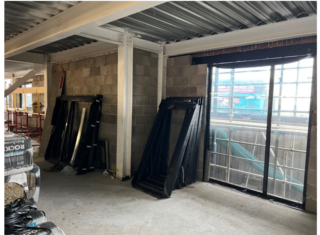
Door / window installation on-going
