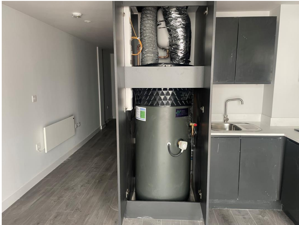
Student Wing – KERS unit installation
