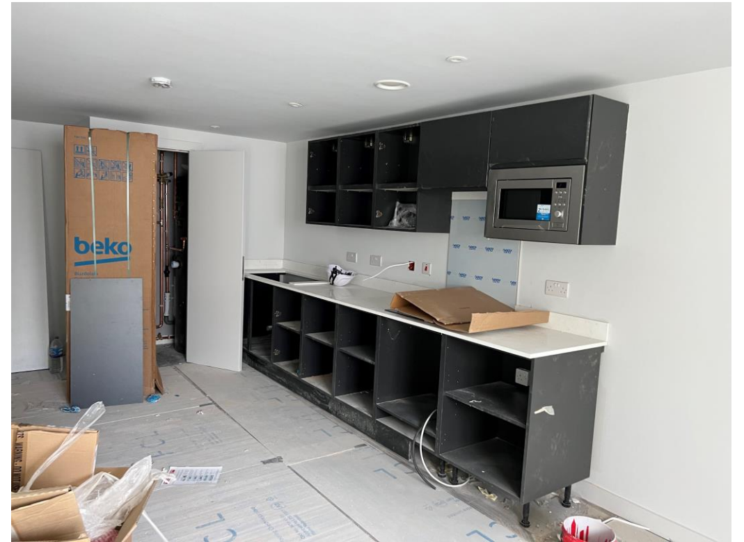
Student Wing – Kitchen installation on-going
