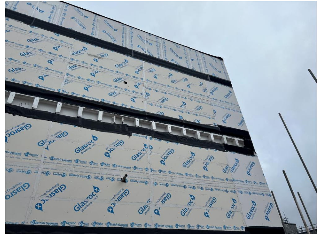
Weather boarding installation
