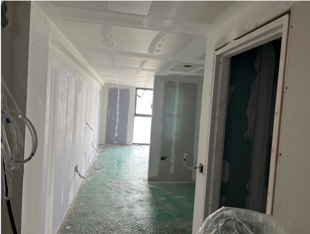
Residential Block – Adhesive screed binder being applied
