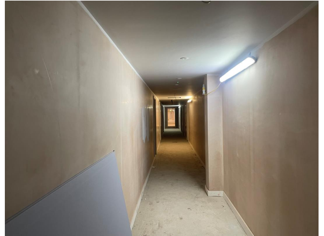
Student Wing – Internal finishes on-going
