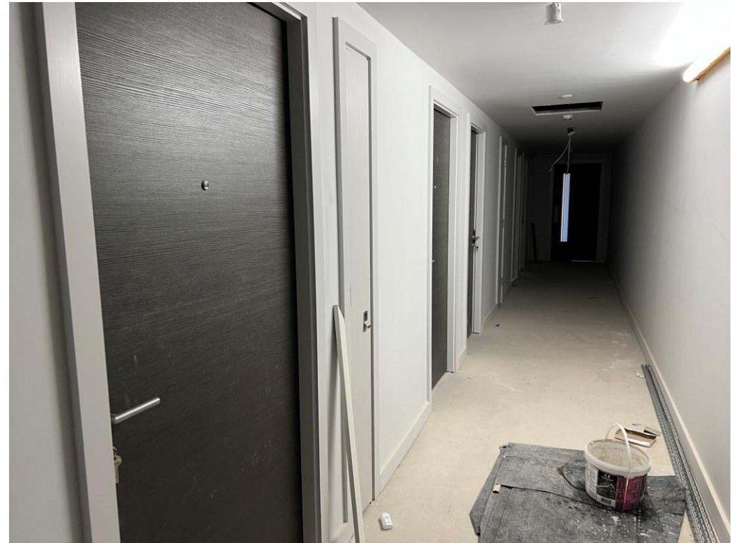
Student Wing – Internal finishes on-going
