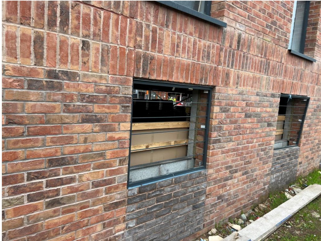
Vent grills installed to undercroft parking area
