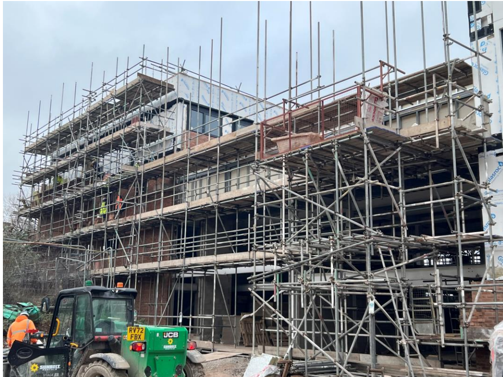
Commercial Block – Brickwork Installation
