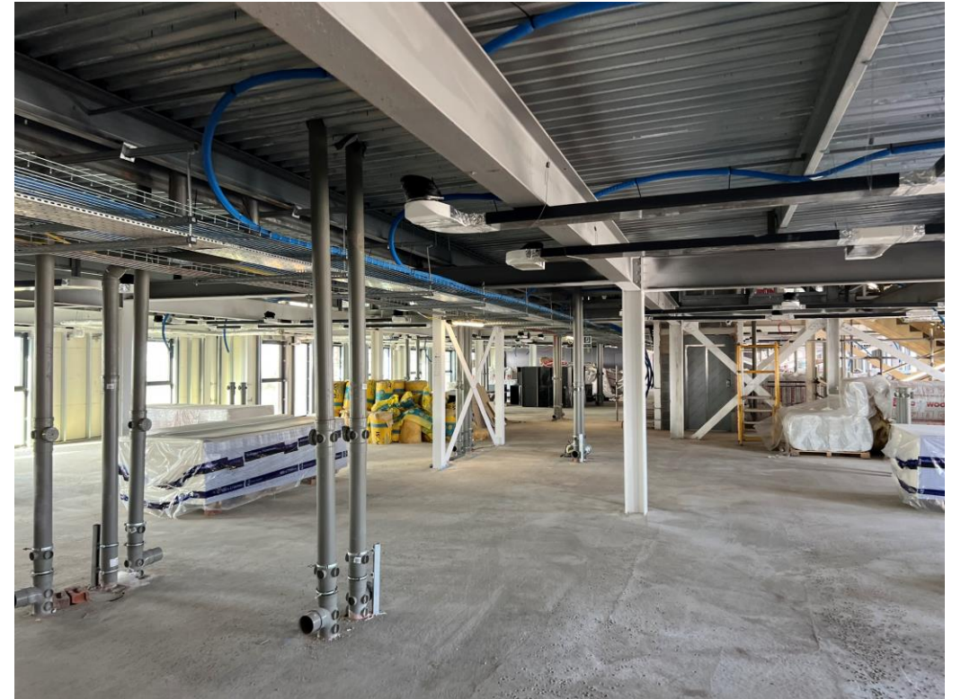
Residential wing – General site activity
