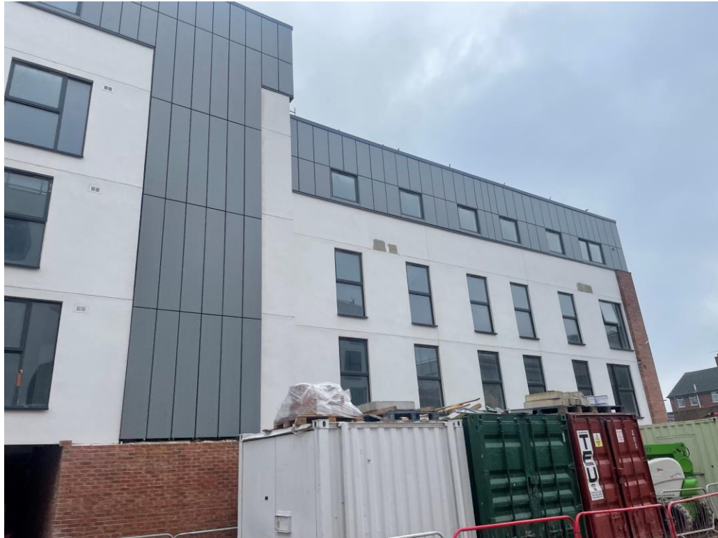
Student Block – Cladding installation complete
