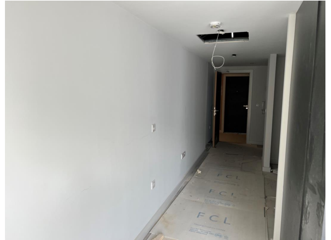
Residential Block – Internal finishes on-going
