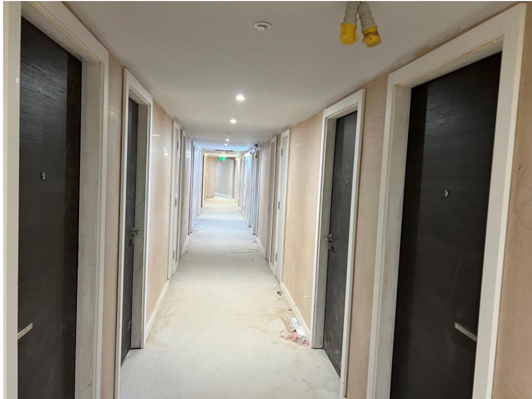
Student Wing – Internal finishes on-going
