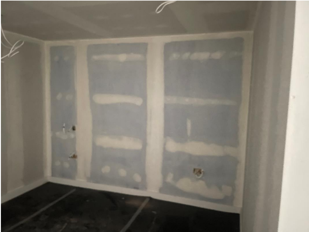
Student Wing – Internal walls boarded, taped and jointed
