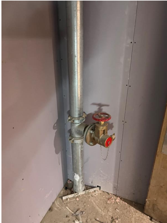
Student Wing – Internal finishes on-going
