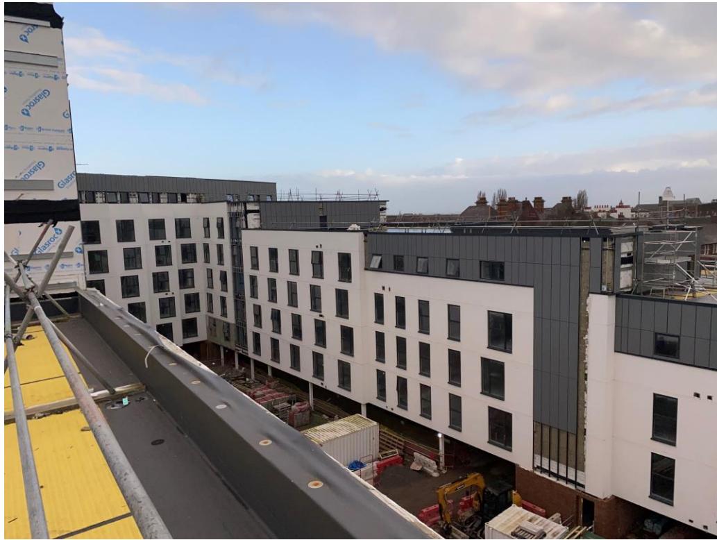
Student Wing – Cladding installation on-going
