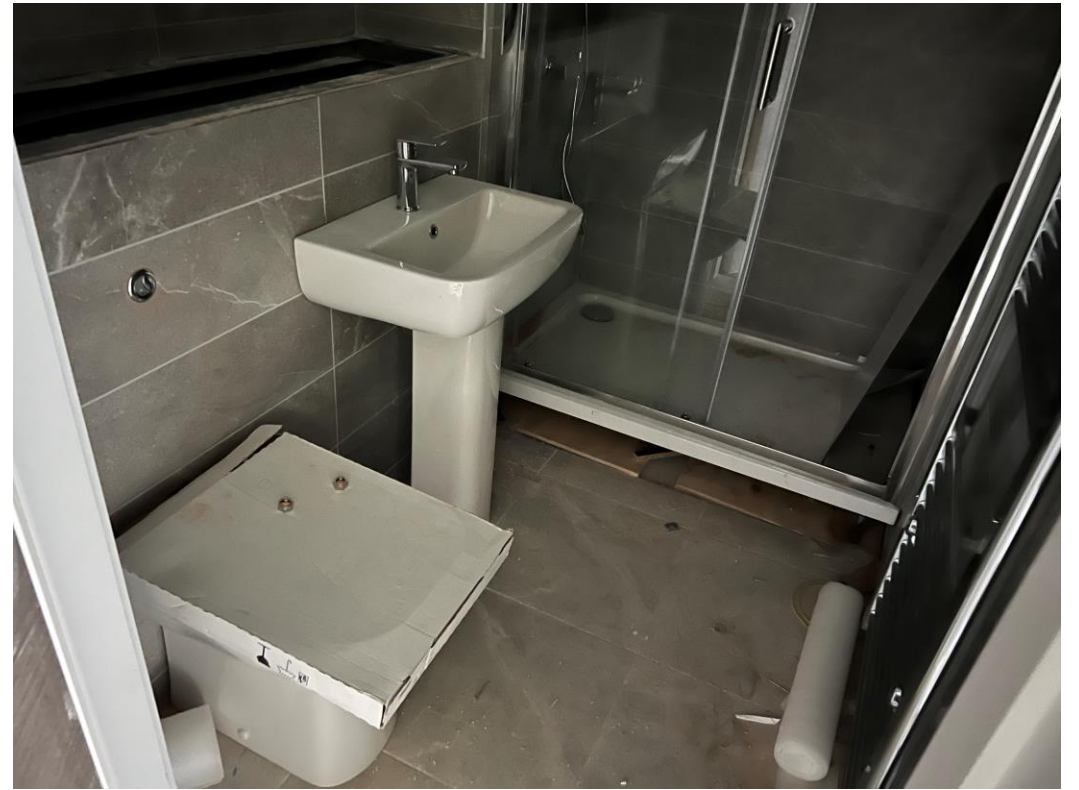
Residential Block – Bathroom appliance installation complete
