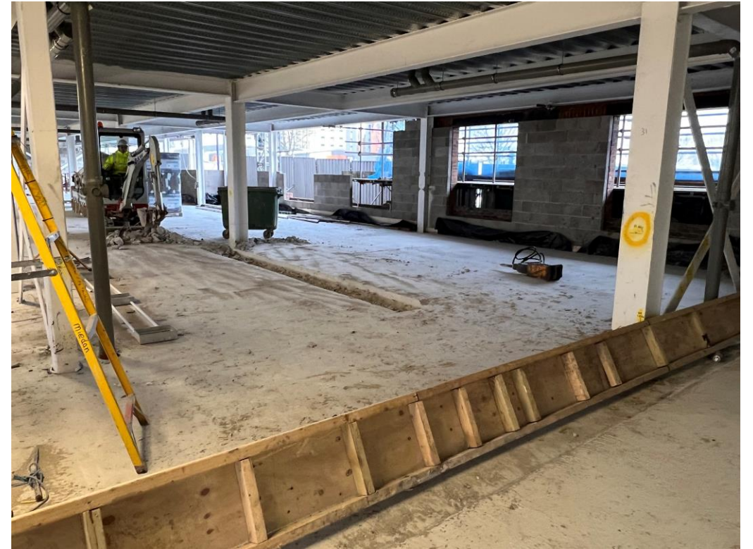
Residential Block – Ground floor concrete slab and drainage alterations
