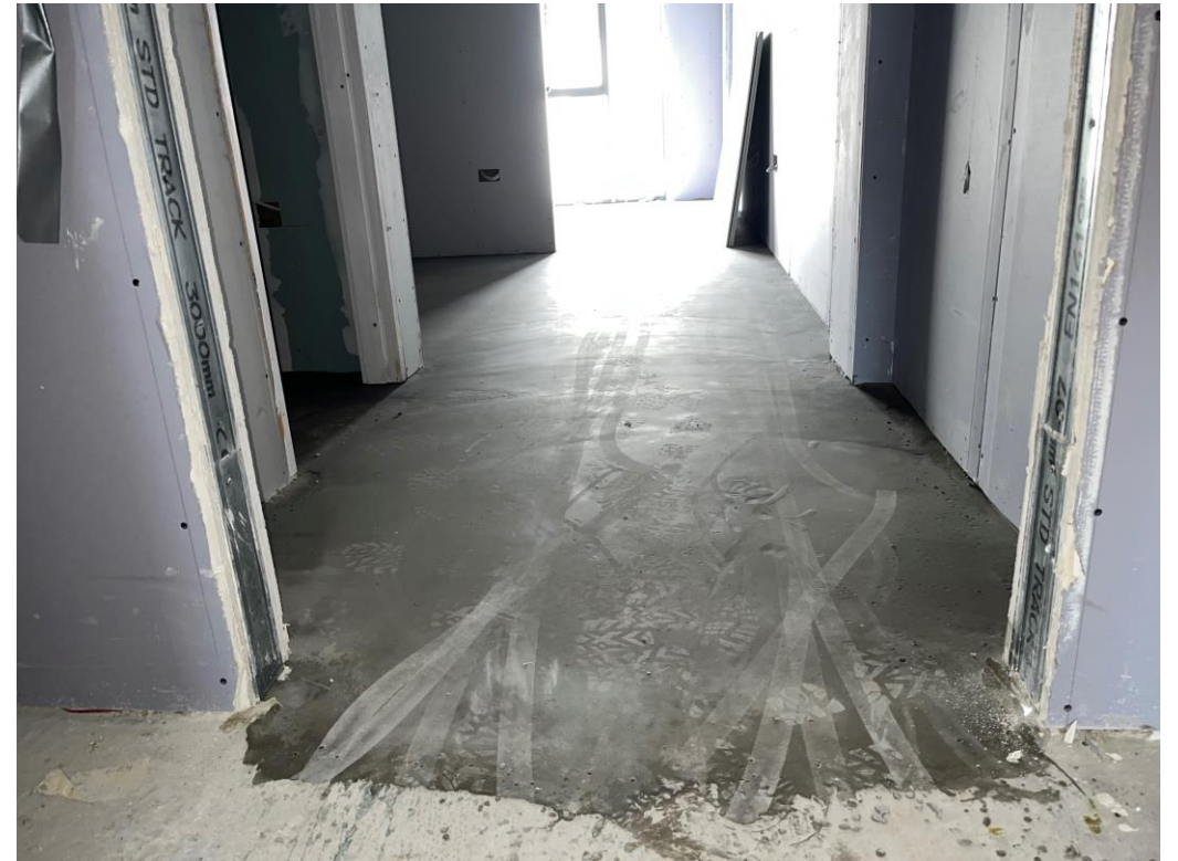
Residential Block – Self-levelling screed on-going
