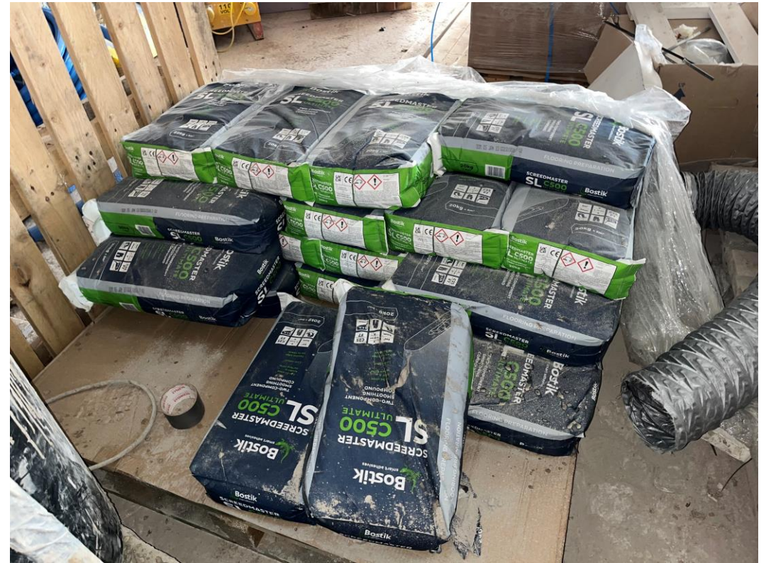
Material Storage – Self-levelling screed
