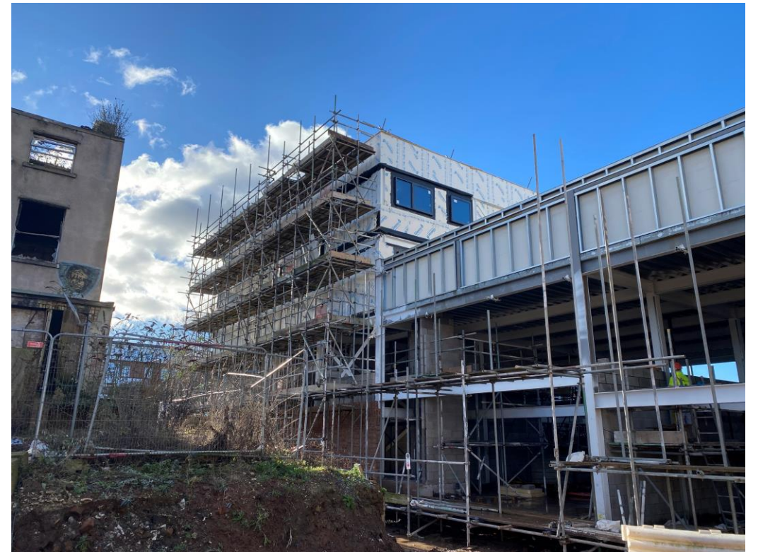
Commercial Block – Scaffolding, SFS and weatherboarding
