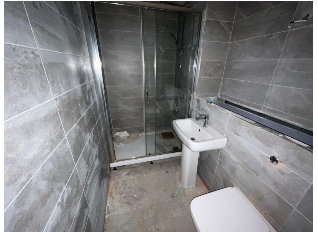
Student Wing – Bathroom appliance installation complete
