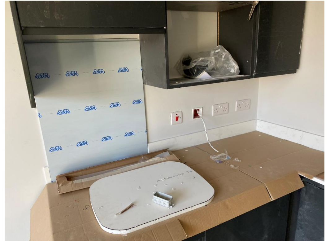
Residential Block – Kitchen sink and splashback installation
