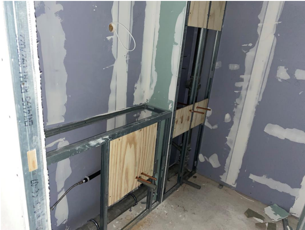
Residential Block – IPS on-going
