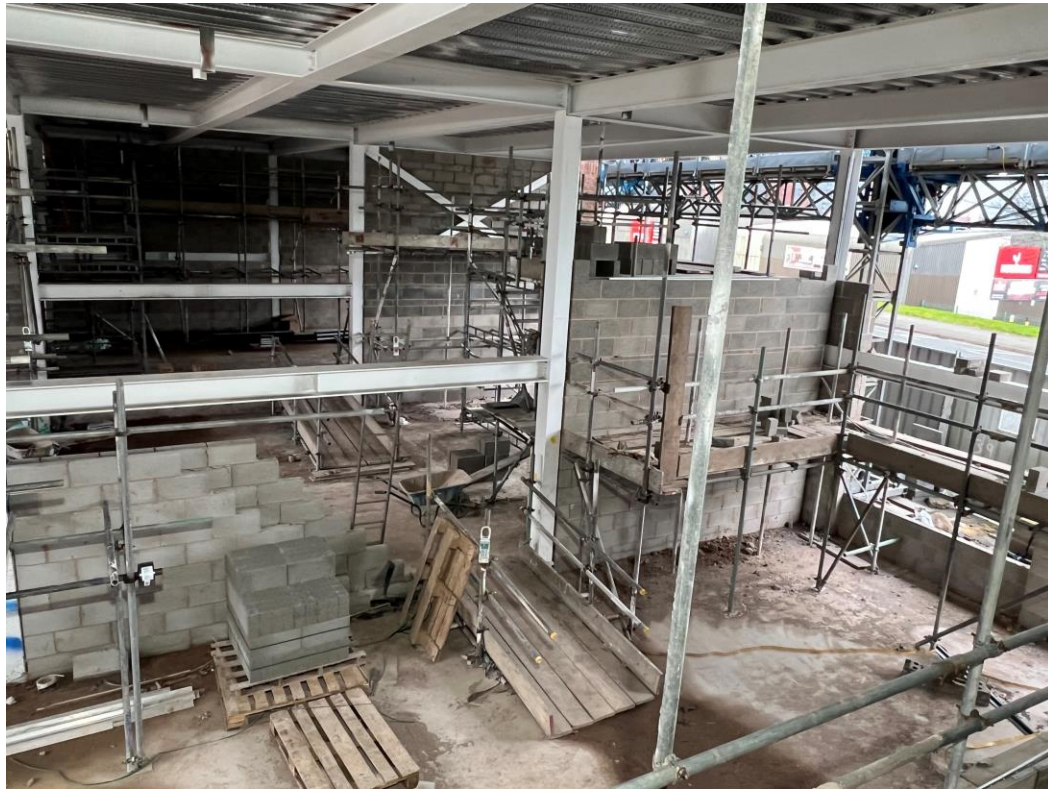
Commercial Block – Internal blockwork on-going
