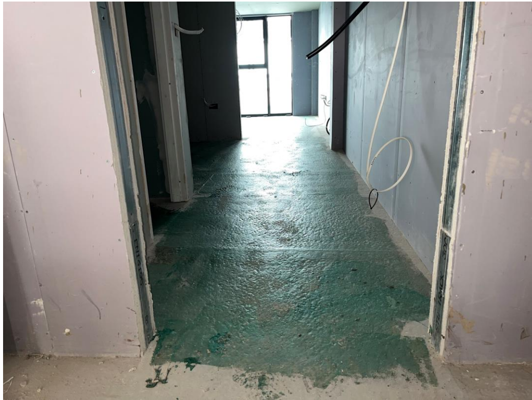
Residential Block – Adhesive screed binder being applied
