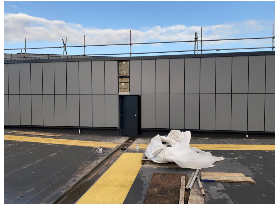
Student Wing – Cladding installation nearing completion
