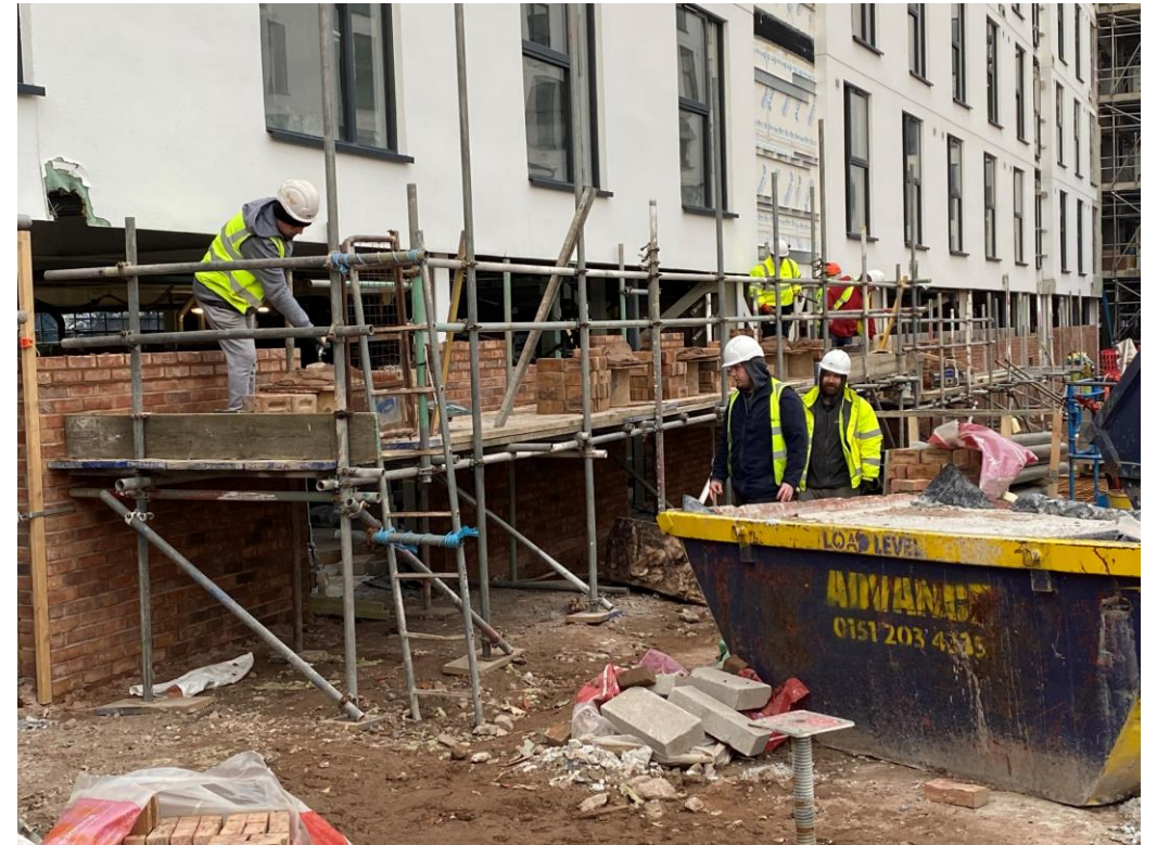
Residential Block – External brickwork on-going
