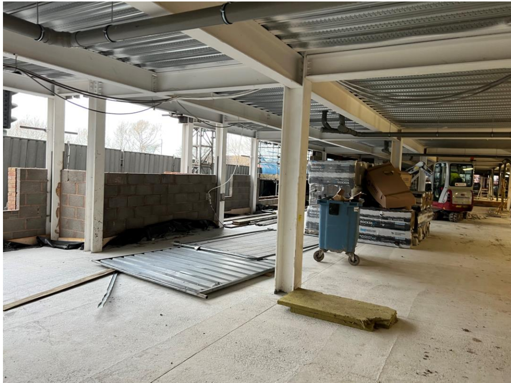
Residential Block – External cavity wall on-going
