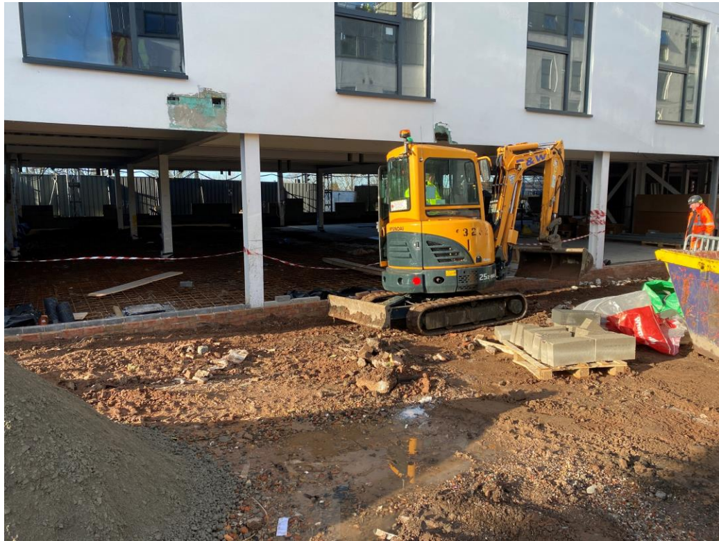
Residential Block – External brickwork on-going
