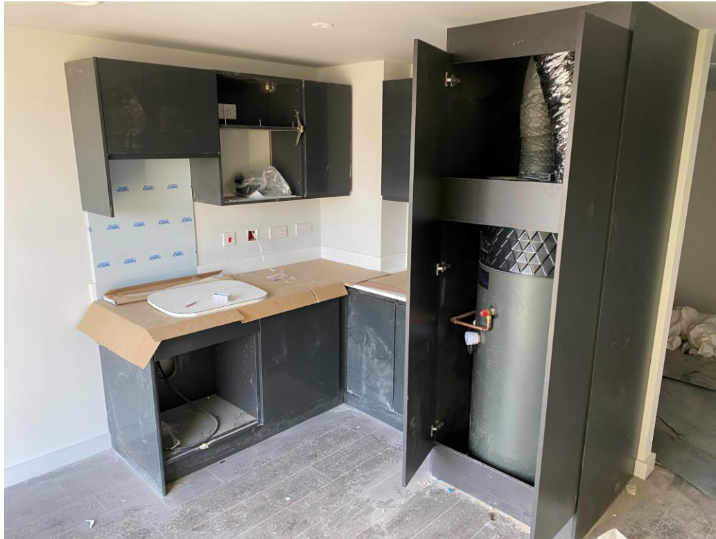
Residential Block – Kitchen installation on-going
