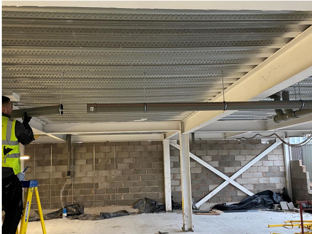
Commercial Block – Internal drainage installation on-going
