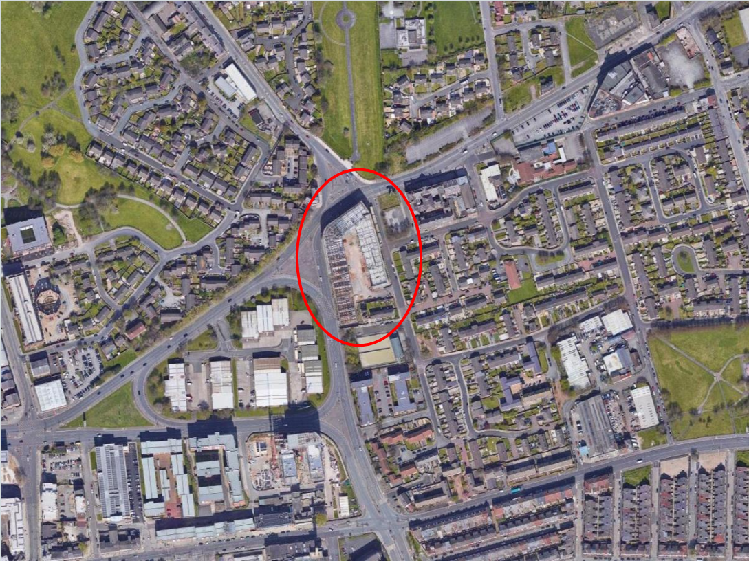
Aerial view of Element – The Quarter site location
