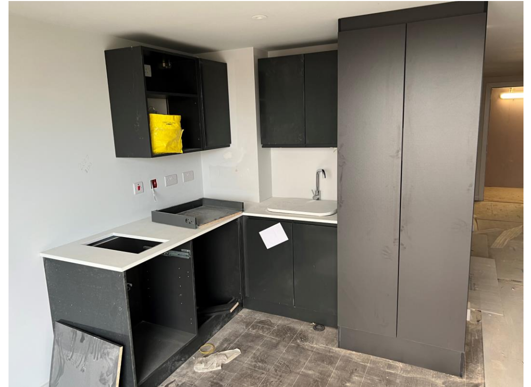
Residential Block – Kitchen installation on-going
