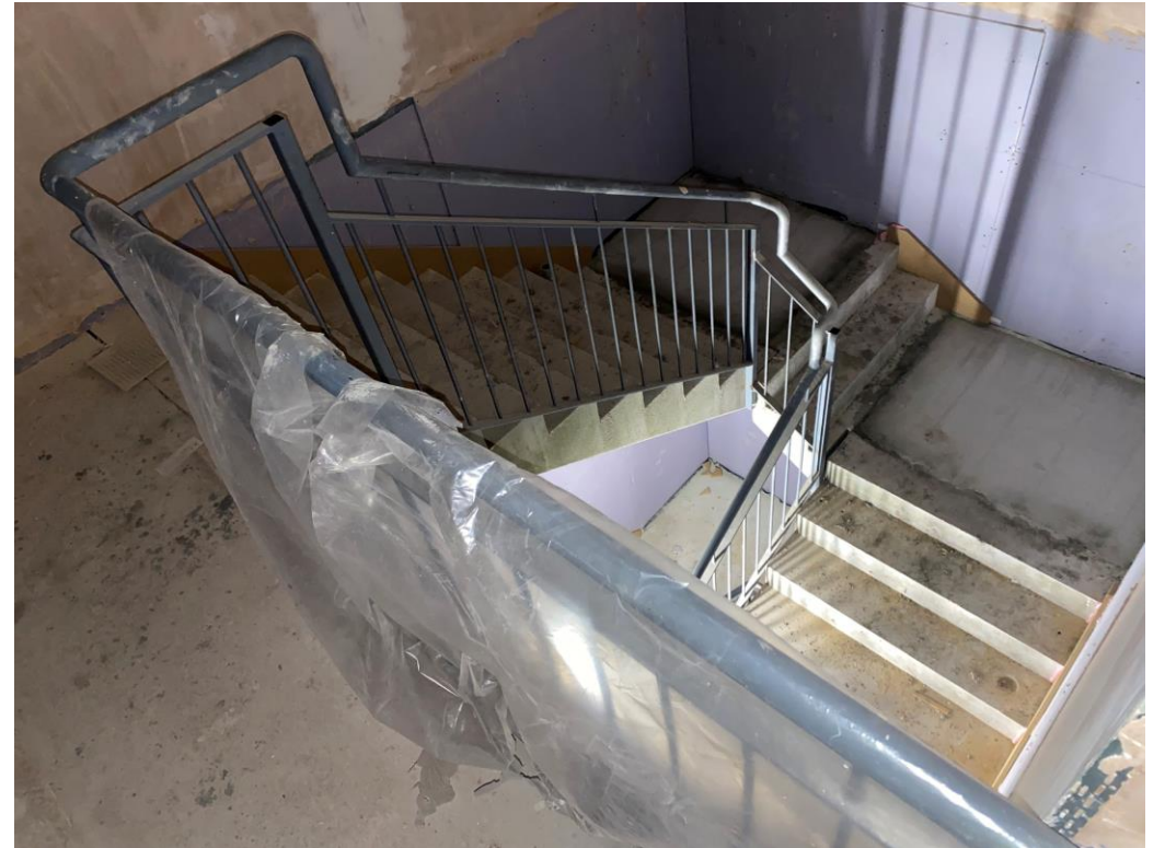
Student Wing – Metal balustrade installation on-going
