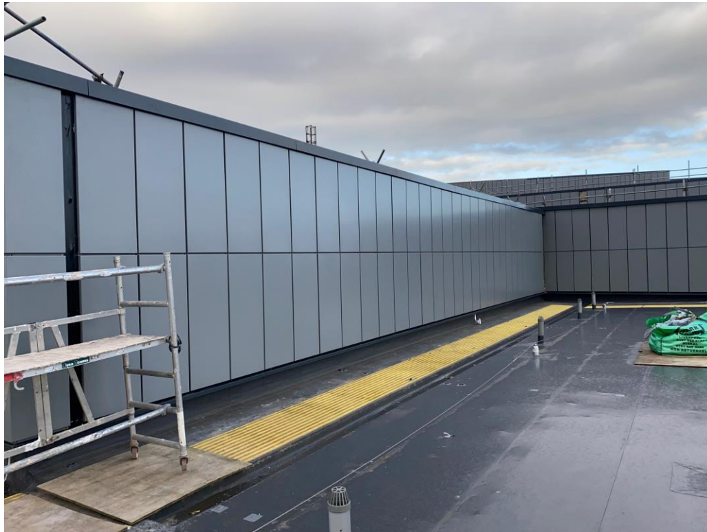
Student Wing – Cladding installation nearing completion
