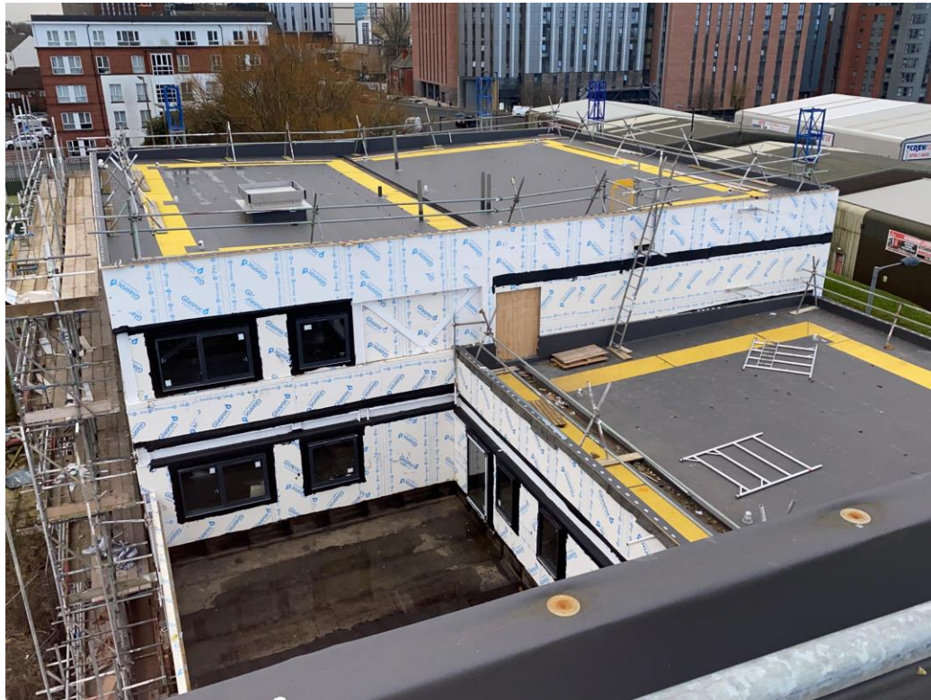
Commercial Block – Mansafe, weatherboarding and edge protection
