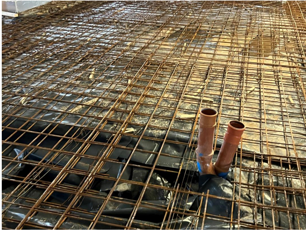
Residential Block – Ground floor slab reinforcement and internal drainage
