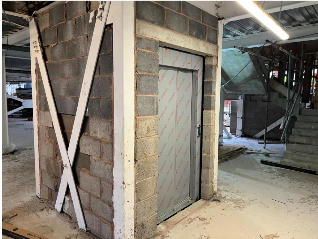
Residential Block – Lift installation
