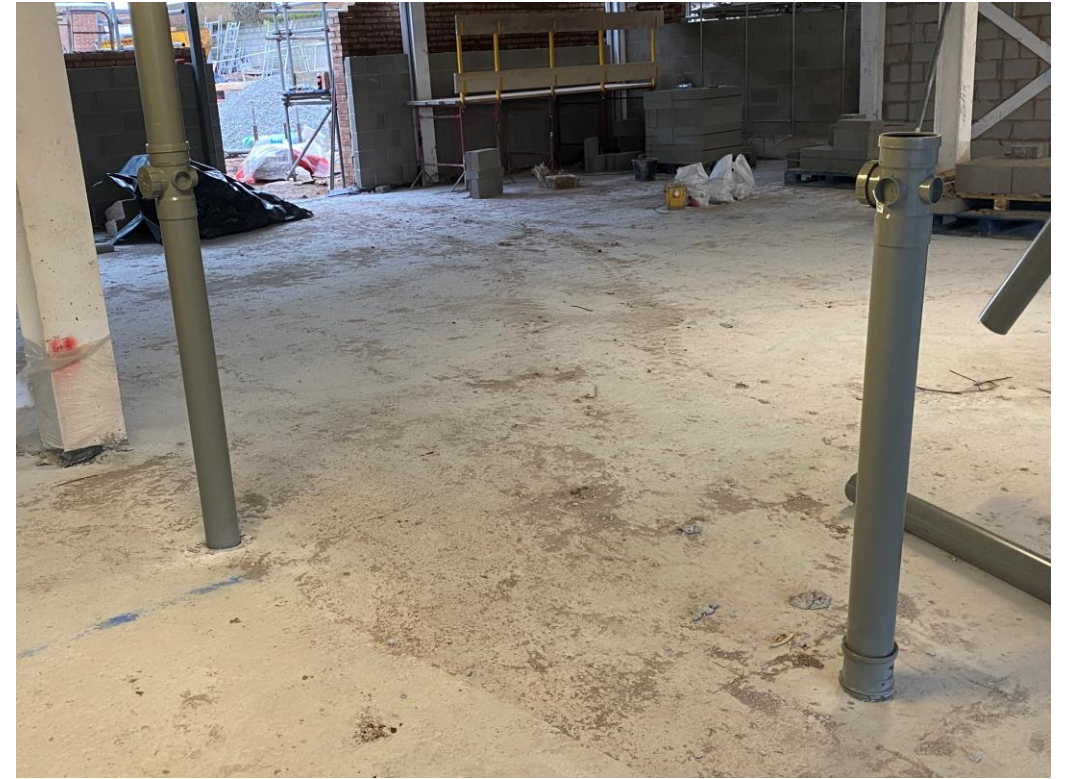
Residential Block – Ground floor slab pour and Internal drainage installation
