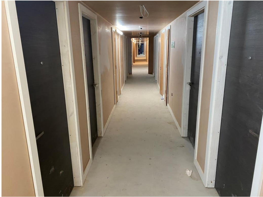
Student Wing – Internal finishes and joinery on-going
