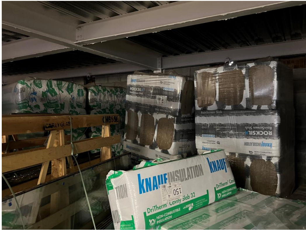
Material Storage – Rocksil insulation
