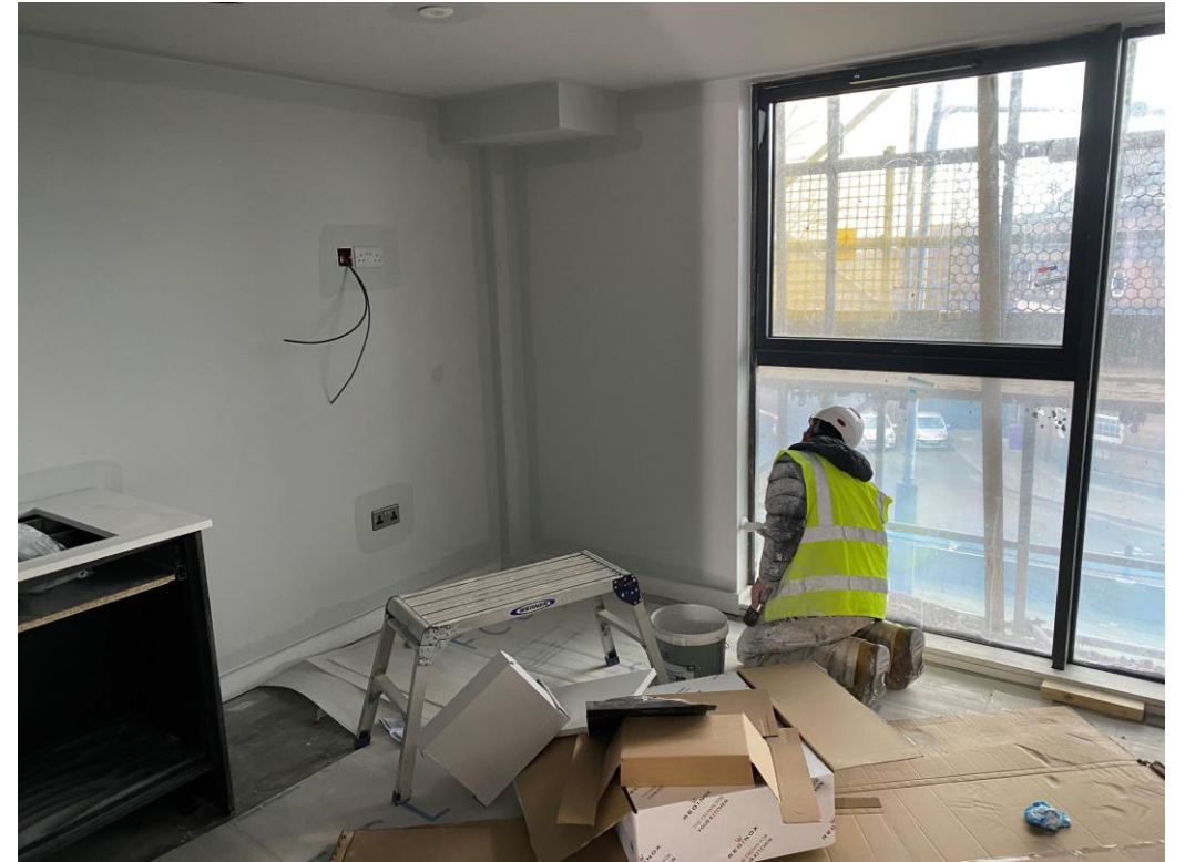
Residential Block - Internal finishes on-going
