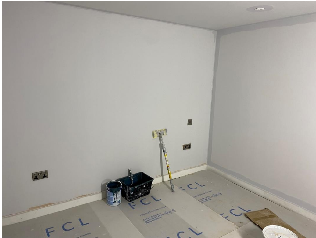
Student Wing – Internal finishes on-going
