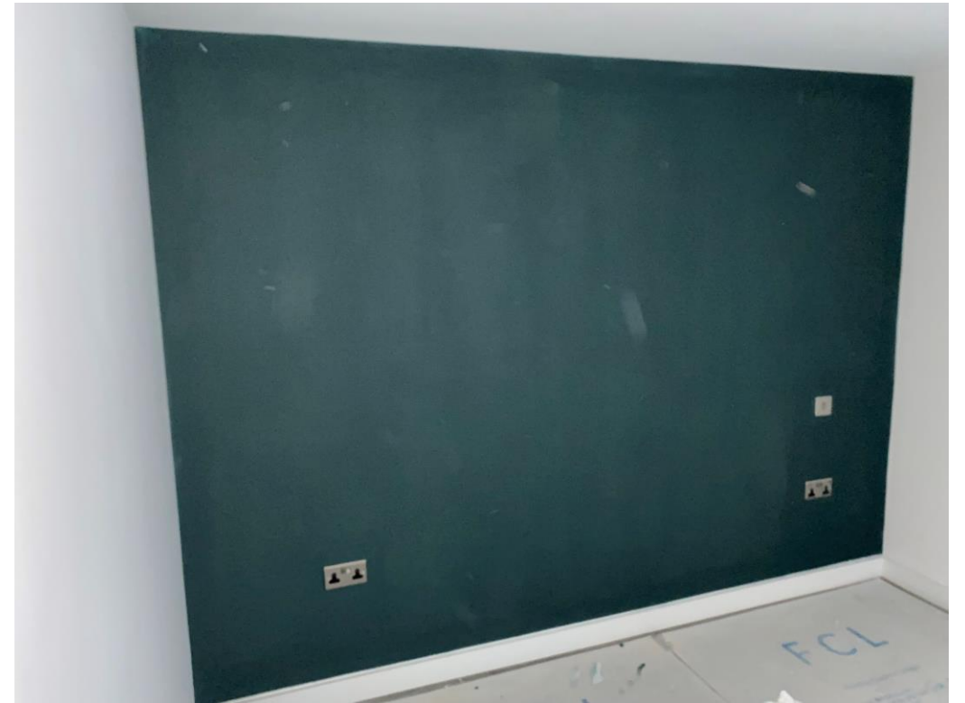
Student Wing – Feature walls to apartments
