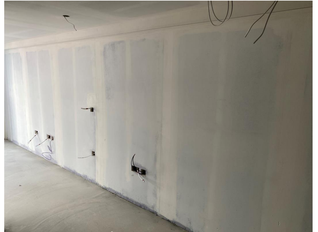
Residential Wing – Internal ceiling and wall mist coat
