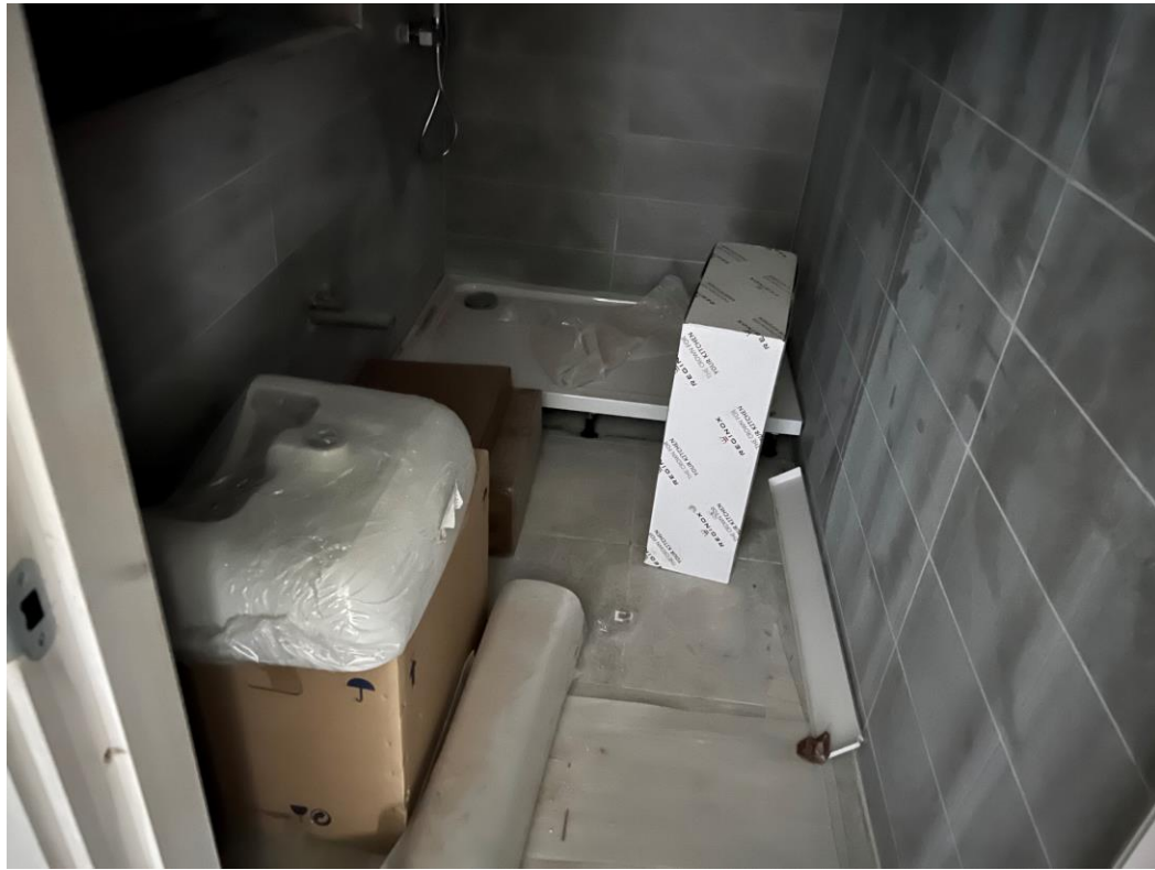
Residential Block – Bathroom appliance installation on-going
