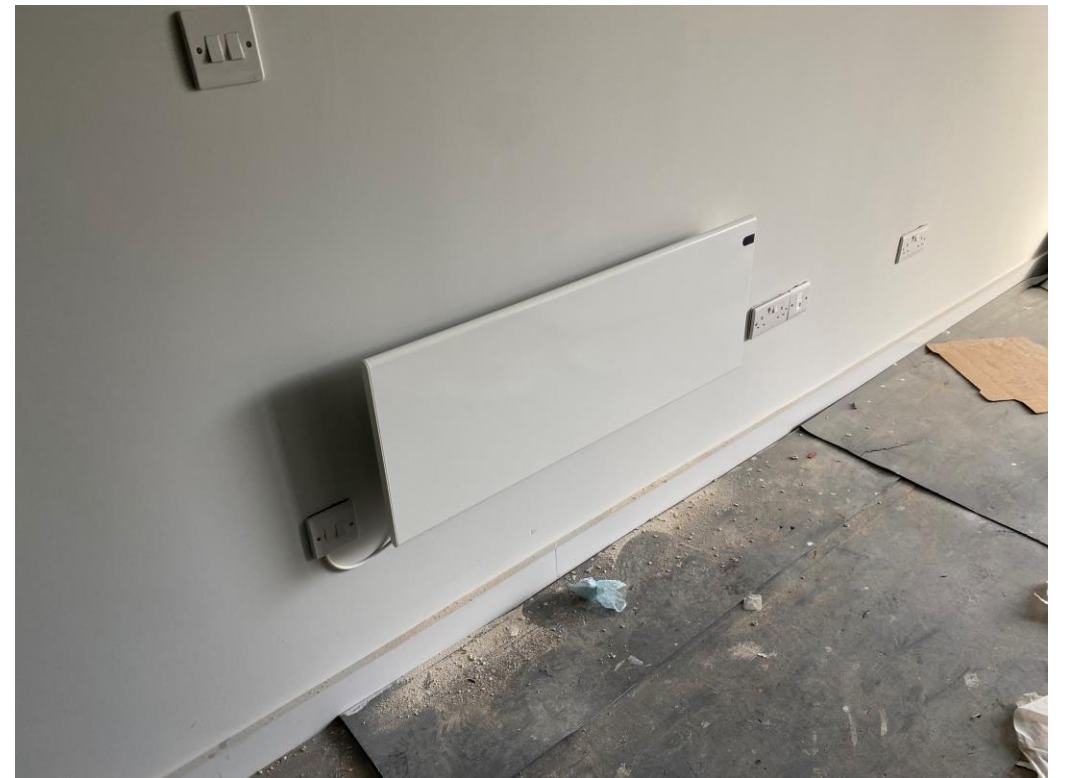
Residential Block – Radiator installation
