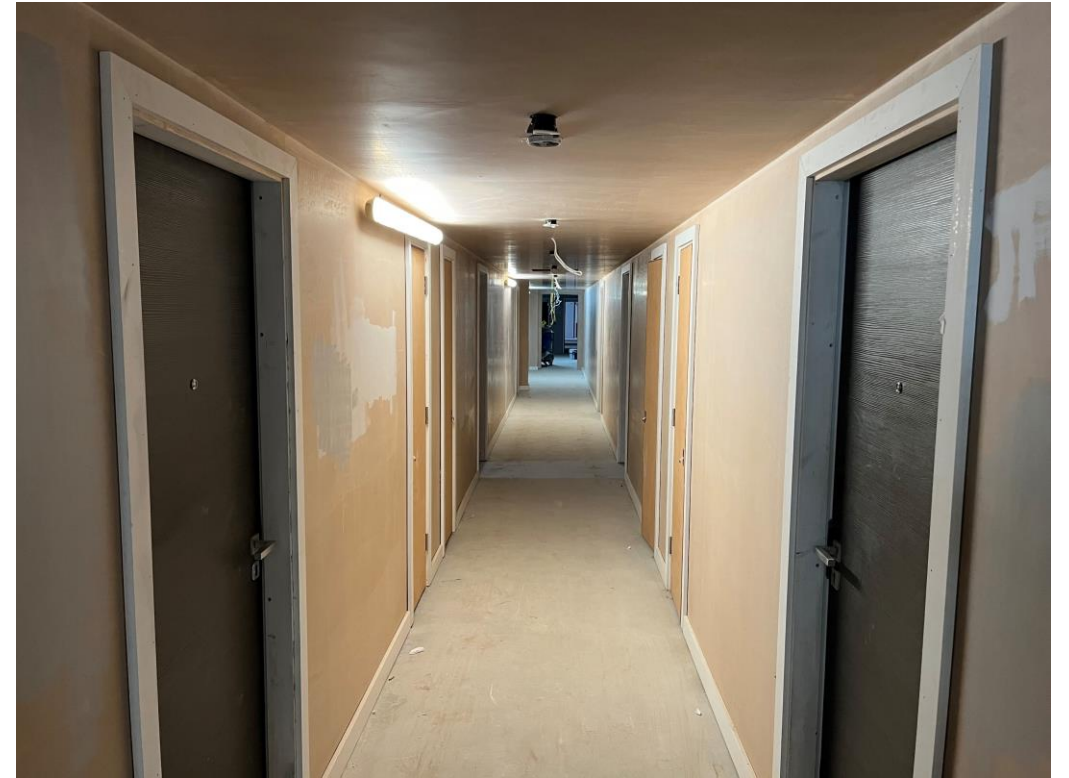
Student Wing – Internal finishes and joinery on-going
