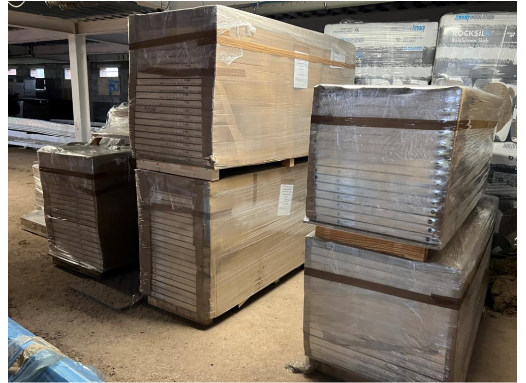
Material storage – Door frames
