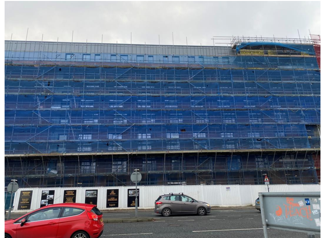
West Derby Road - Site view
