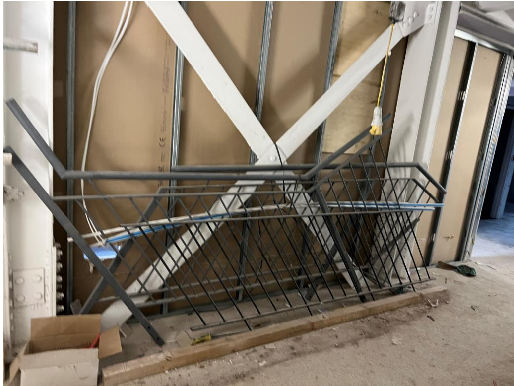
Residential Block – Metal balustrade ready for installation
