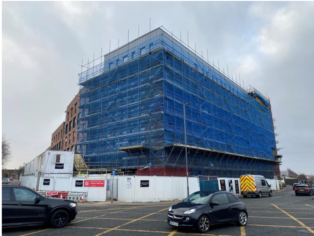
West Derby Road - Site view
