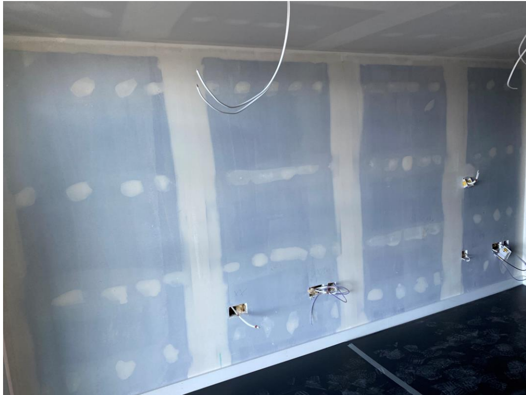
Residential Wing – Internal walls boarded, taped and jointed
