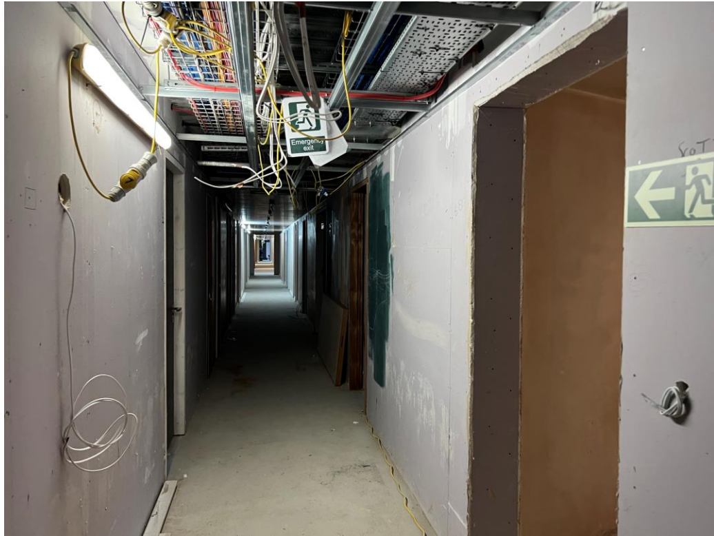
Student Wing – 1 st fix electrical installation on-going
