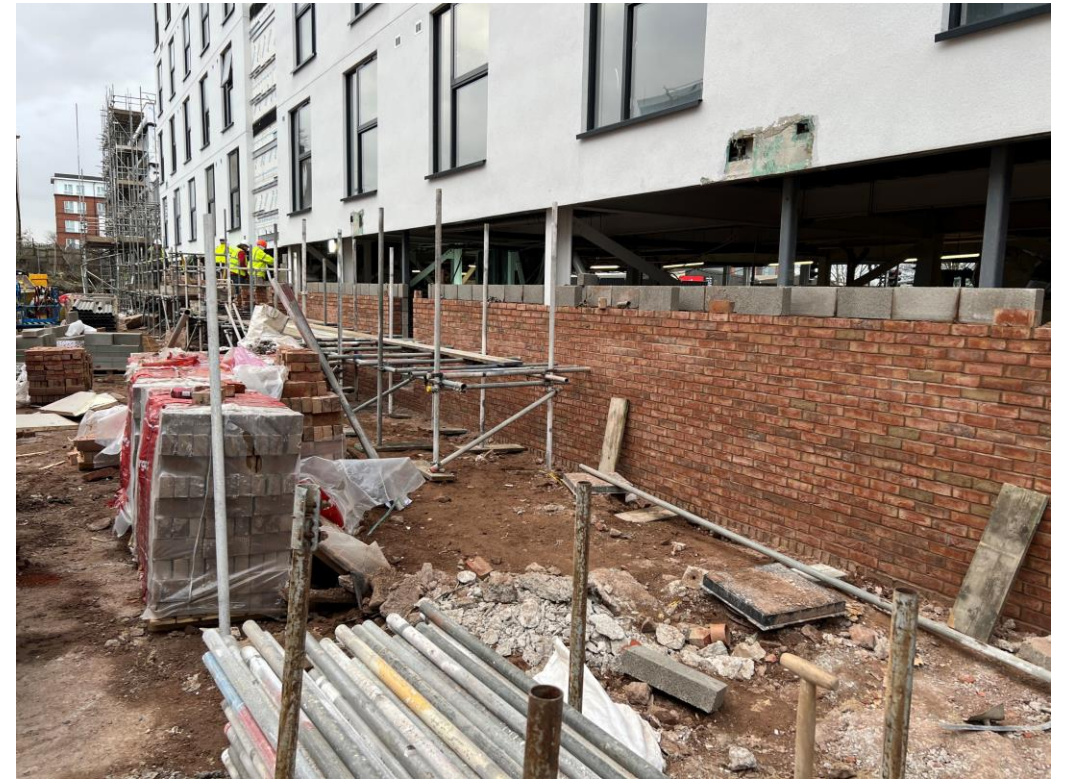
Residential Block – External brickwork on-going
