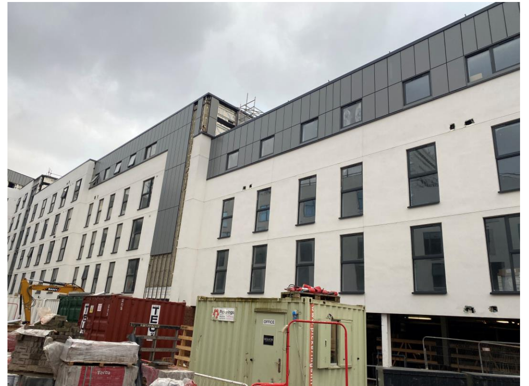
Student Wing – Cladding installation on-going
