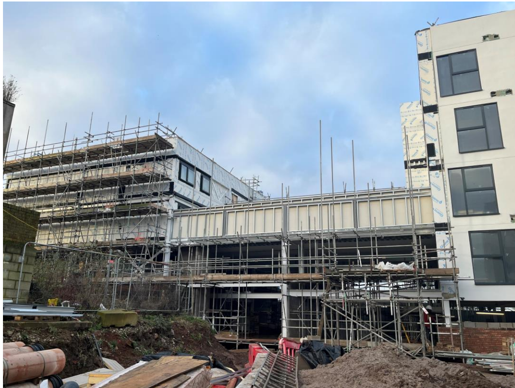
Commercial Block – Scaffolding, SFS and weatherboarding
