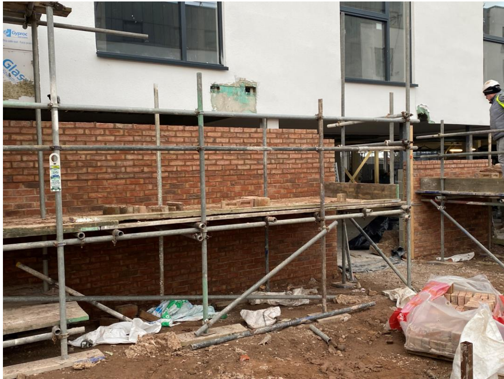
Residential Block – External brickwork on-going
