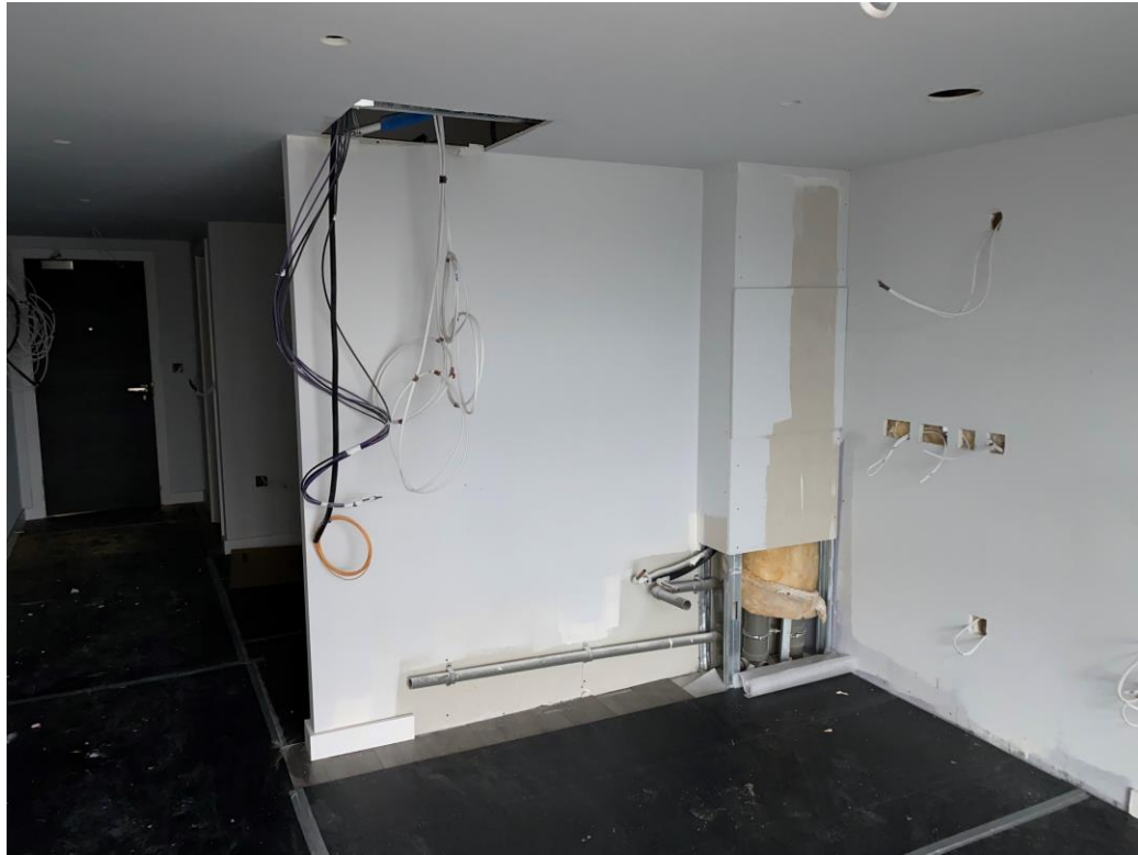
Residential Block - Internal finishes on-going
