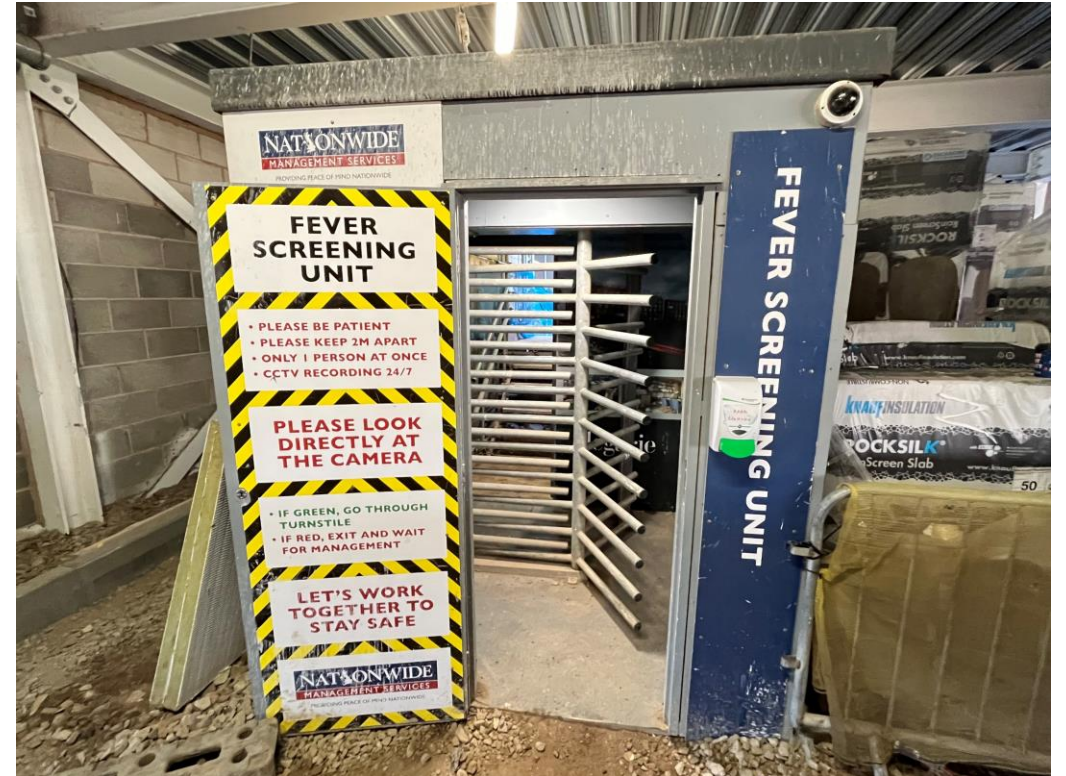
Turnstile being utilised
