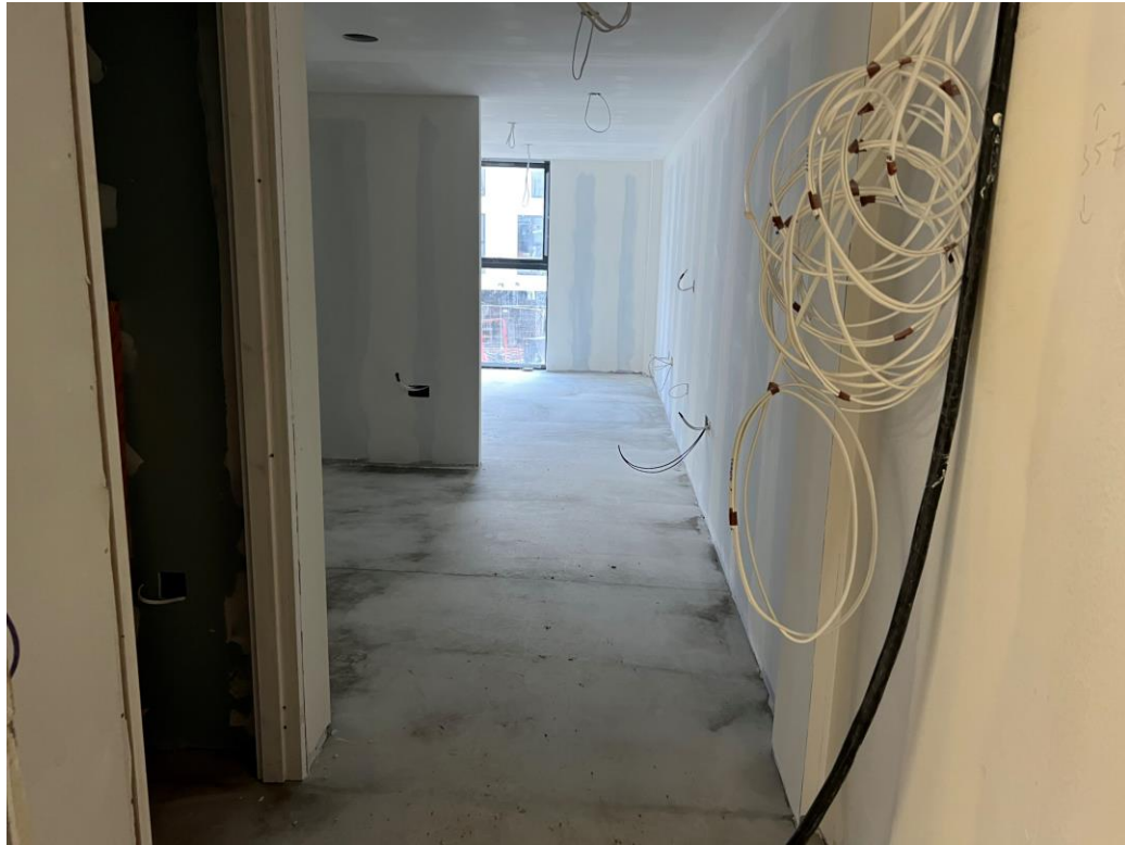
Student Block - Internal finishes on-going
