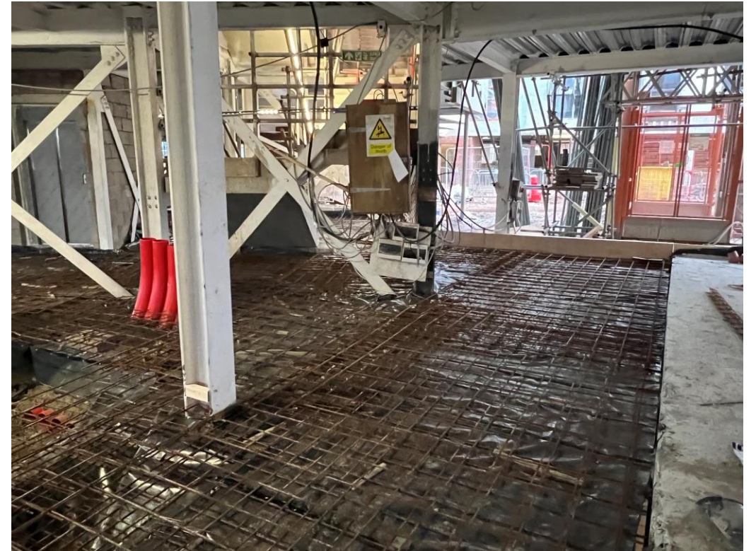
Residential Wing – Ground floor slab reinforcement installation
