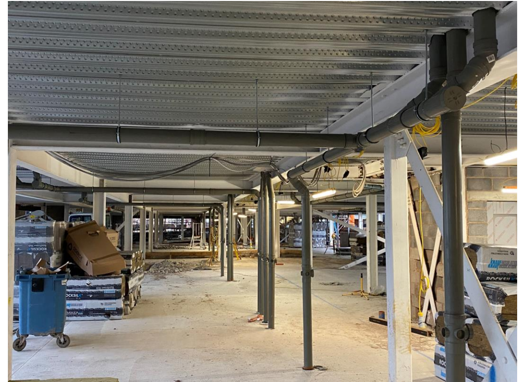
Residential Wing – Internal drainage installation on-going
