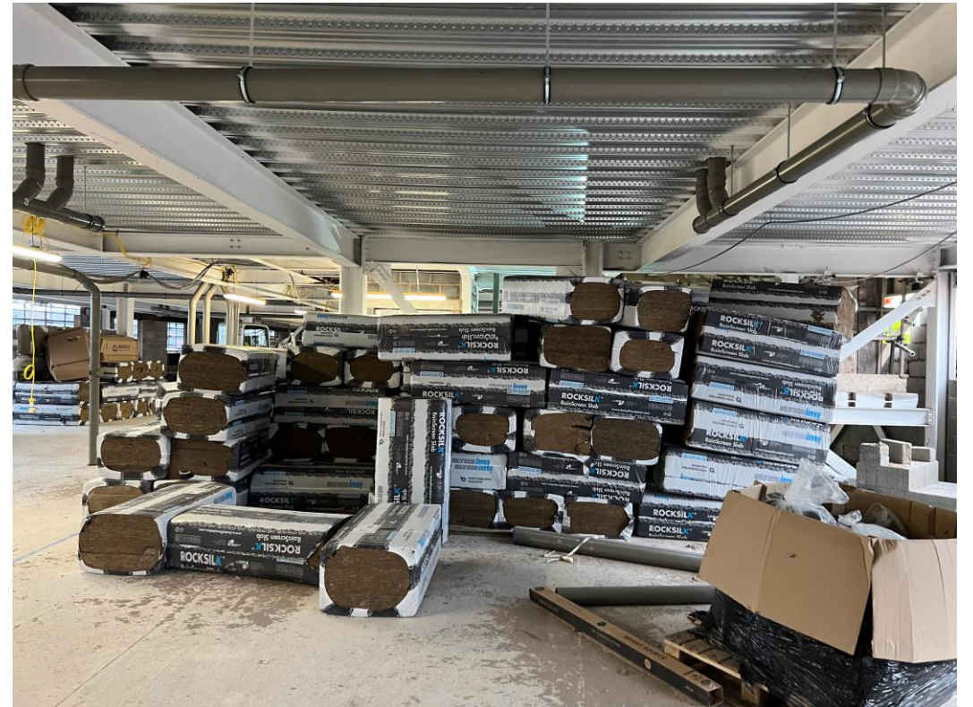
Material Storage – Rocksil insulation
