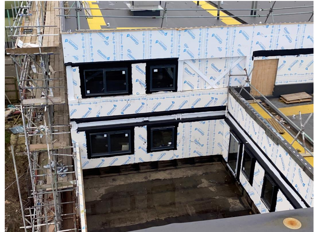
Commercial Block – Mansafe, weatherboarding and edge protection
