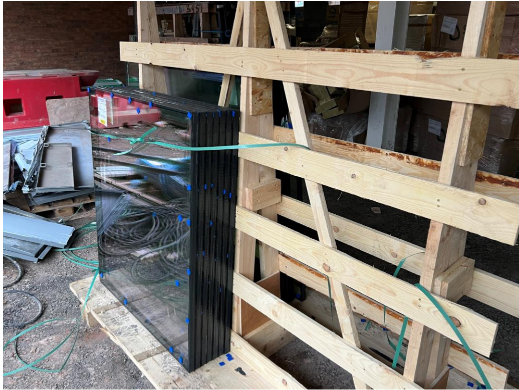
Material storage – Window units
