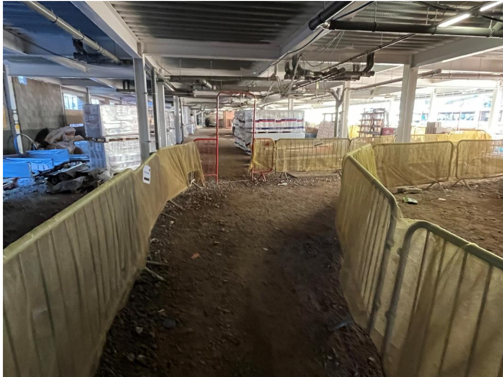
Site segregation in place
