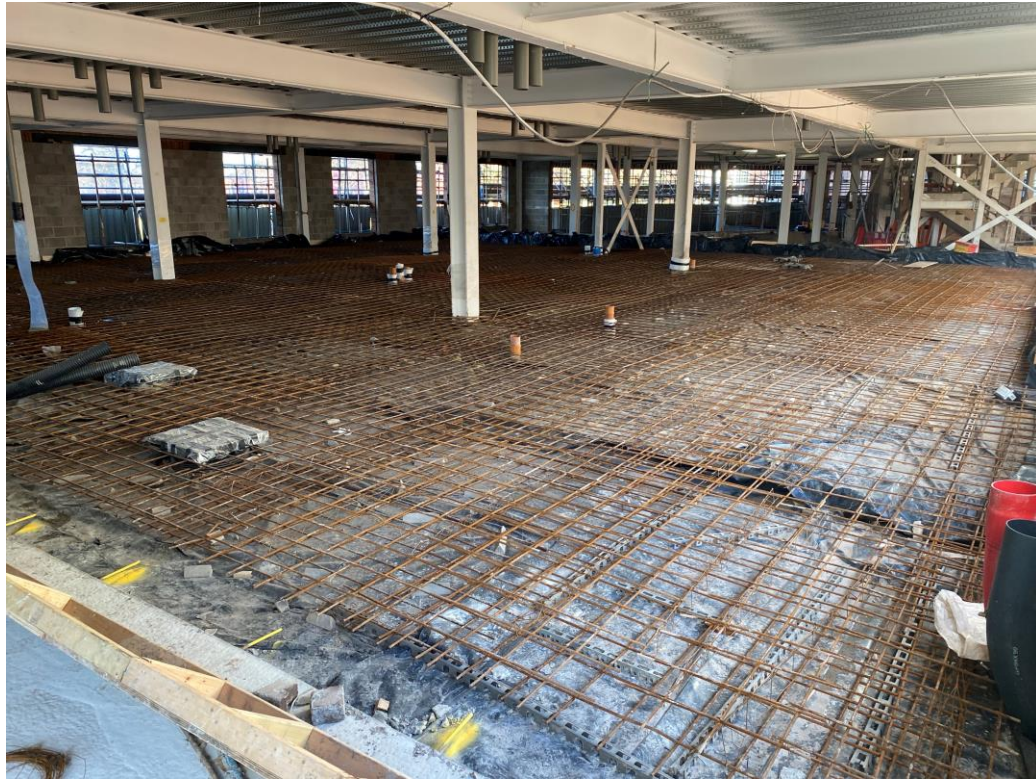
Residential Wing – Ground floor slab reinforcement installation
