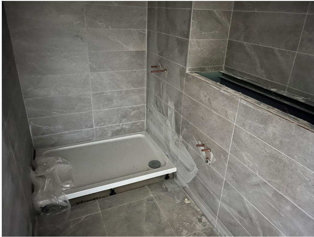
Student Wing – Bathroom appliance installation on-going
