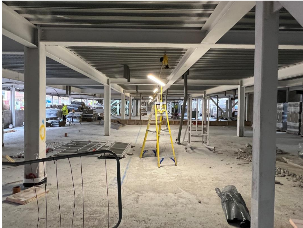
Residential Block – Ground floor concrete slab
