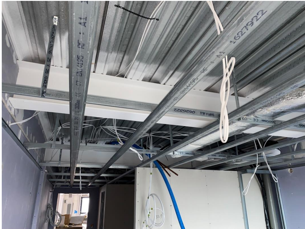
Residential Block – 1 st fix electrical installation and metal ceiling on-going
