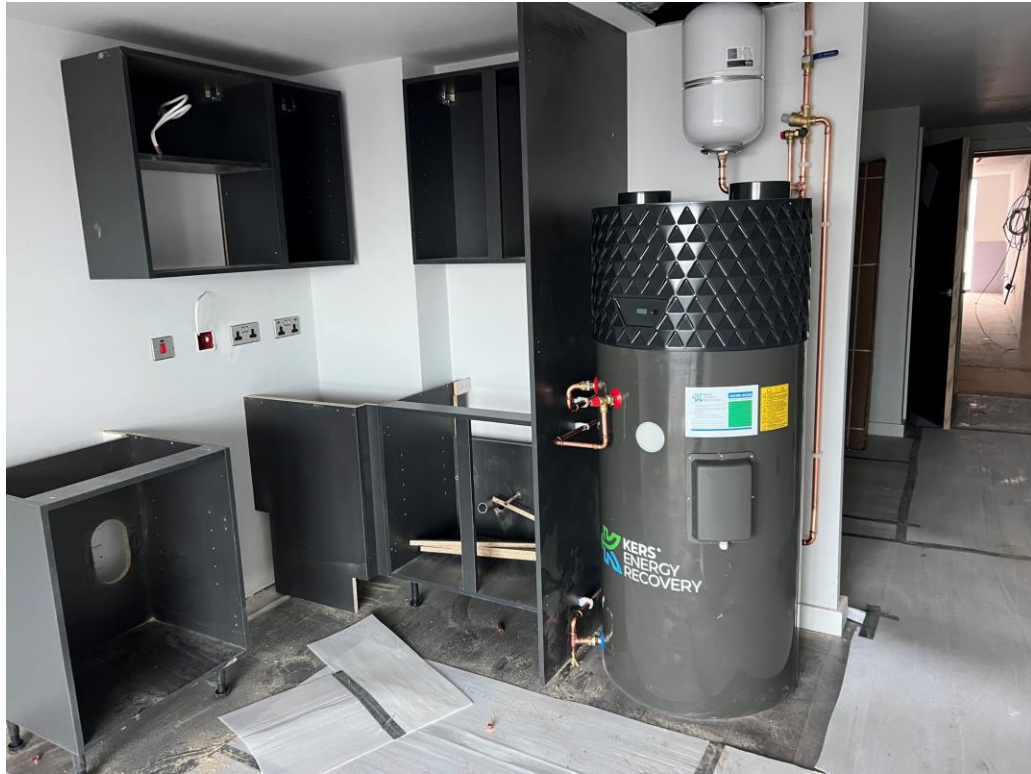
Residential Block – Kitchen installation on-going
