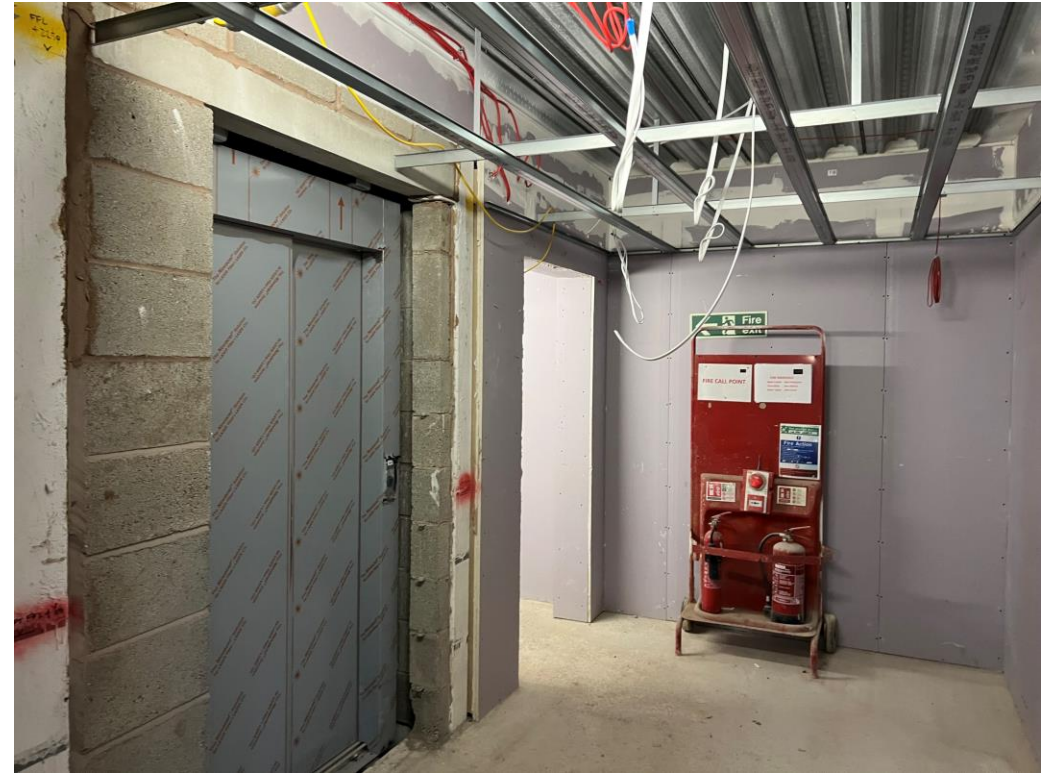
Residential Block – Lift installation
