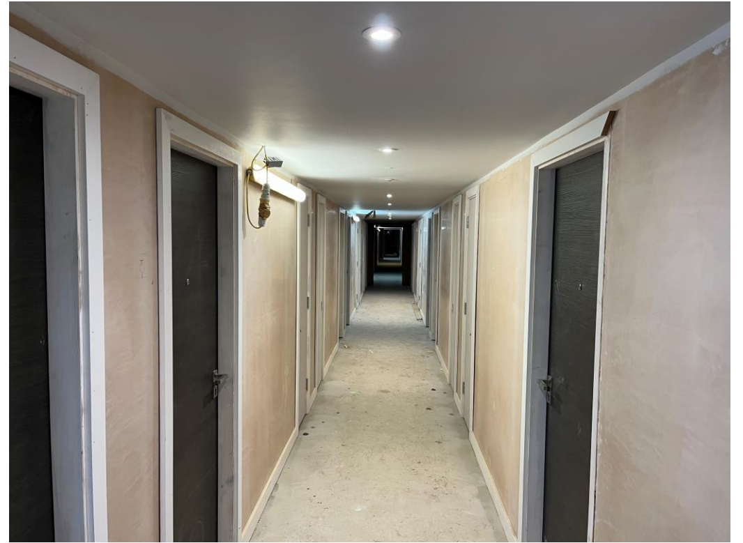
Student Wing – Internal finishes and joinery on-going
