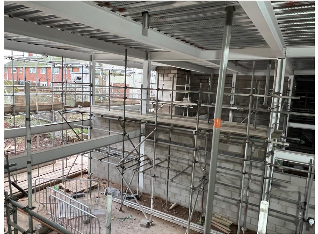
Commercial Block– Internal blockwork on-going
