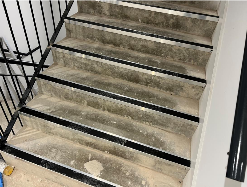
Stair Core – protective nosing's
