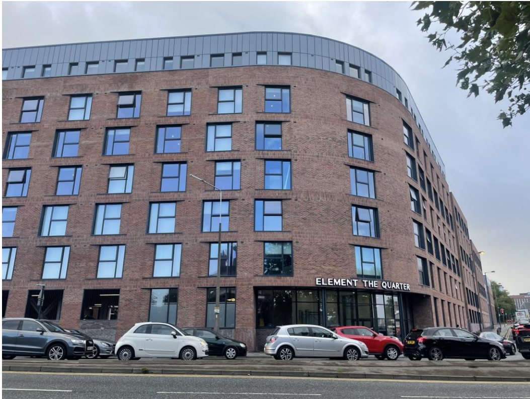
Brunswick Road – Building signage complete
