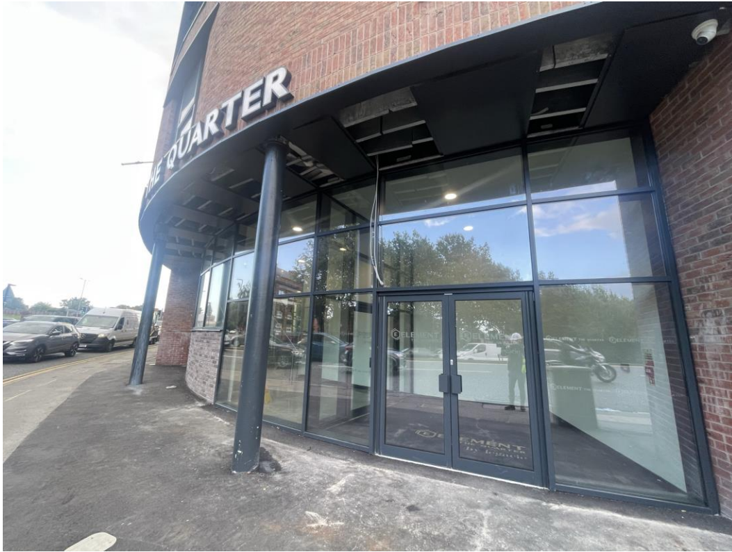
Main Entrance – Curtain Walling
