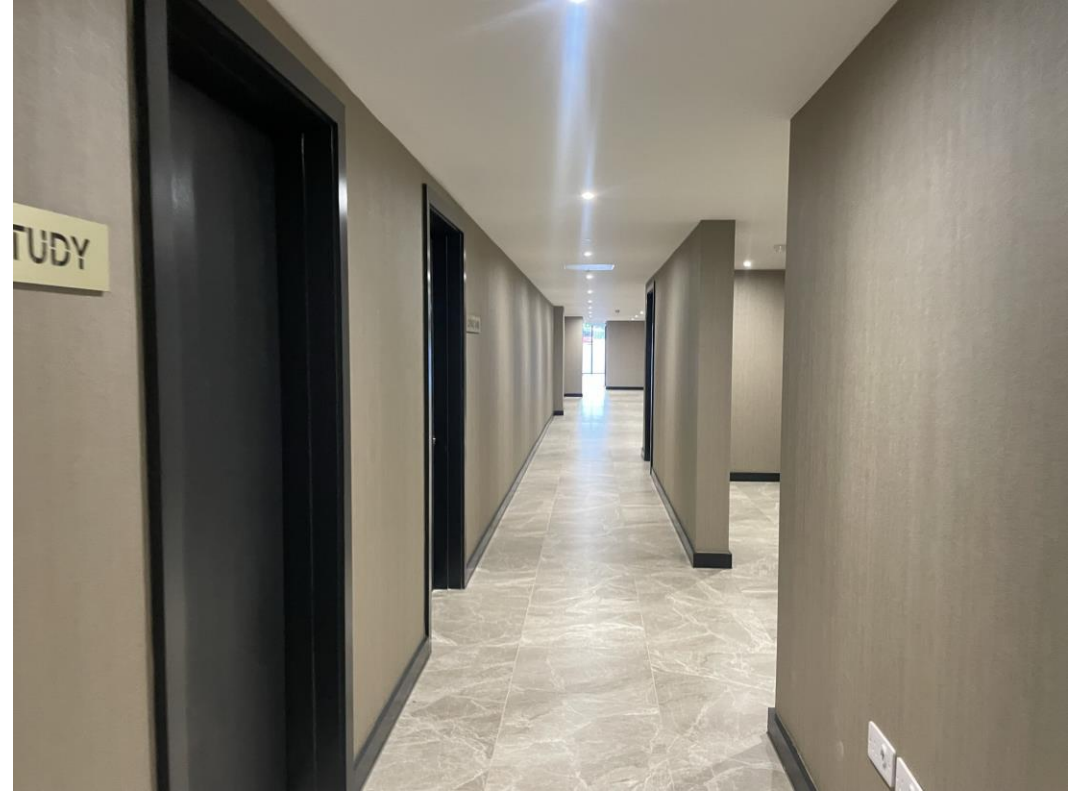
Ground Floor – Corridor finishes
