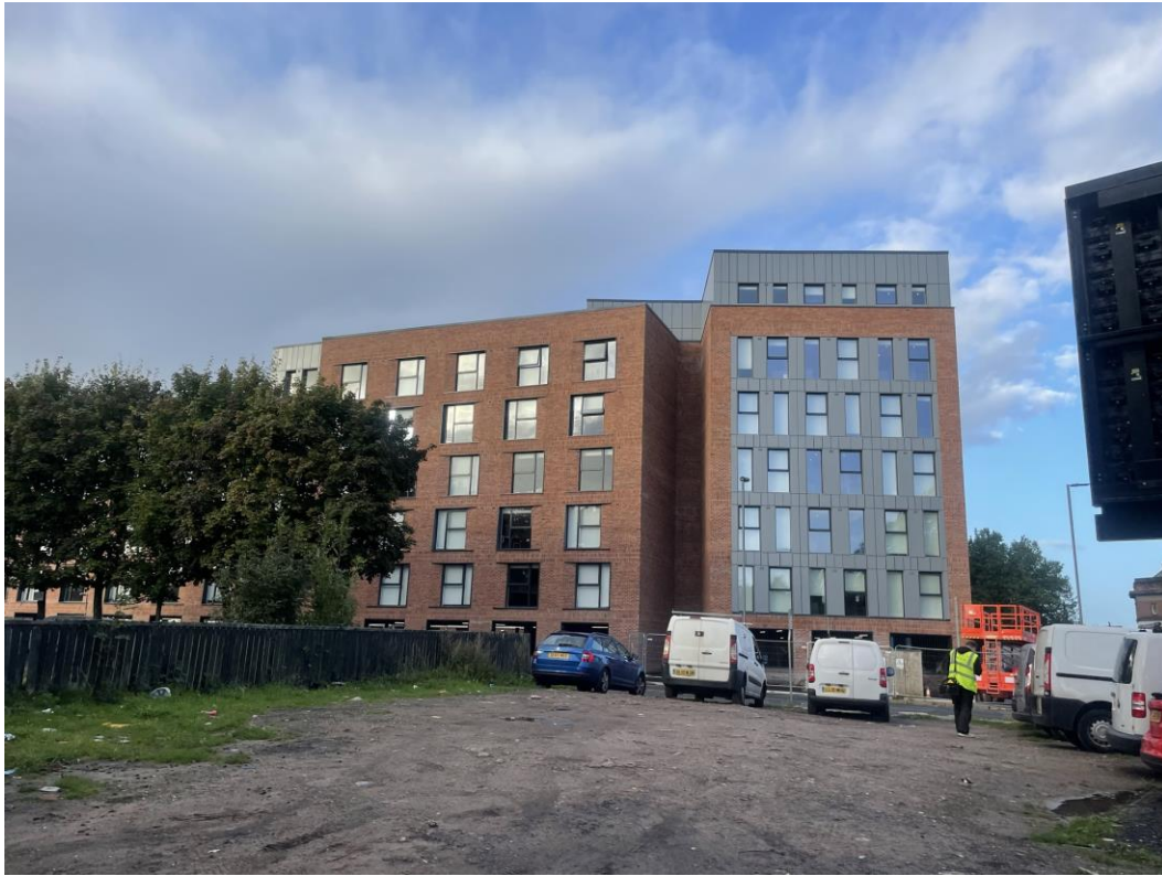
West Derby Road - Site view
