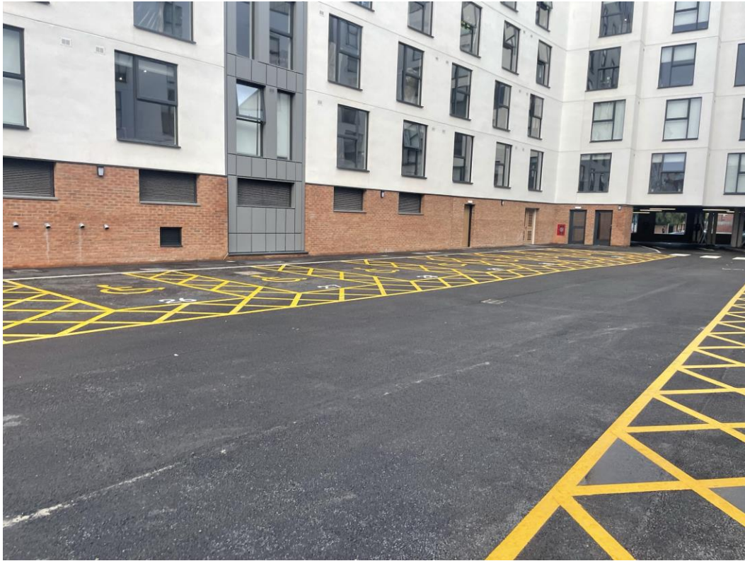
Accessible parking bays
