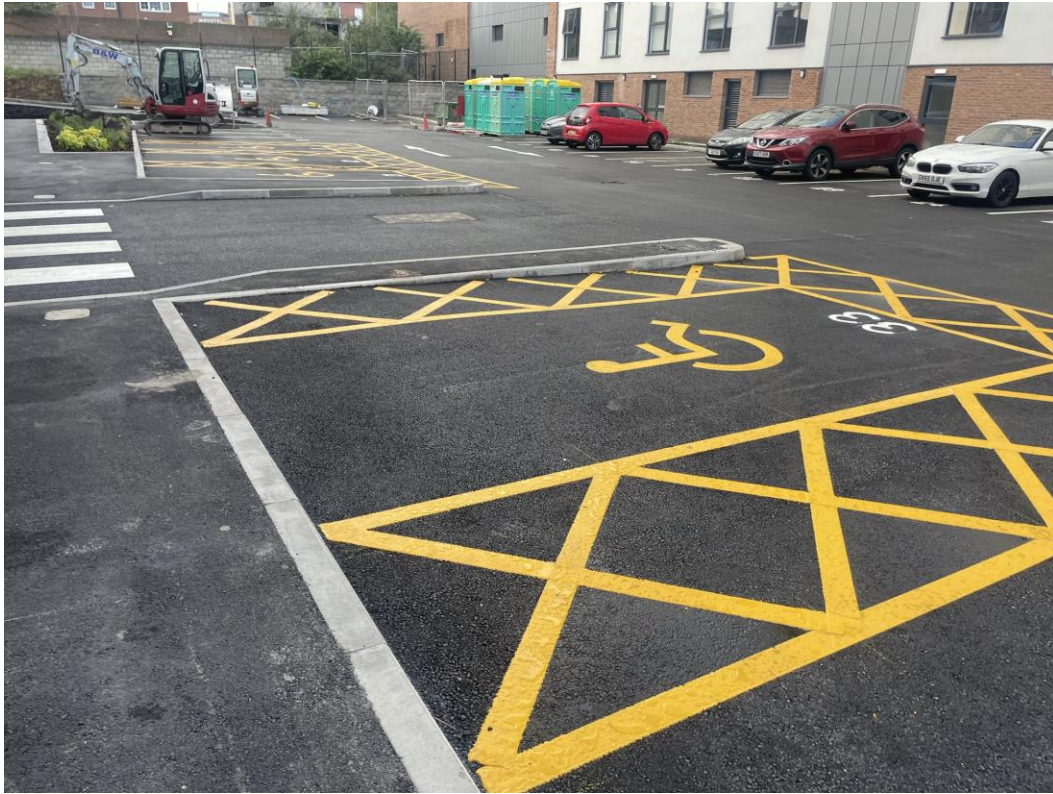
Accessible parking bays
