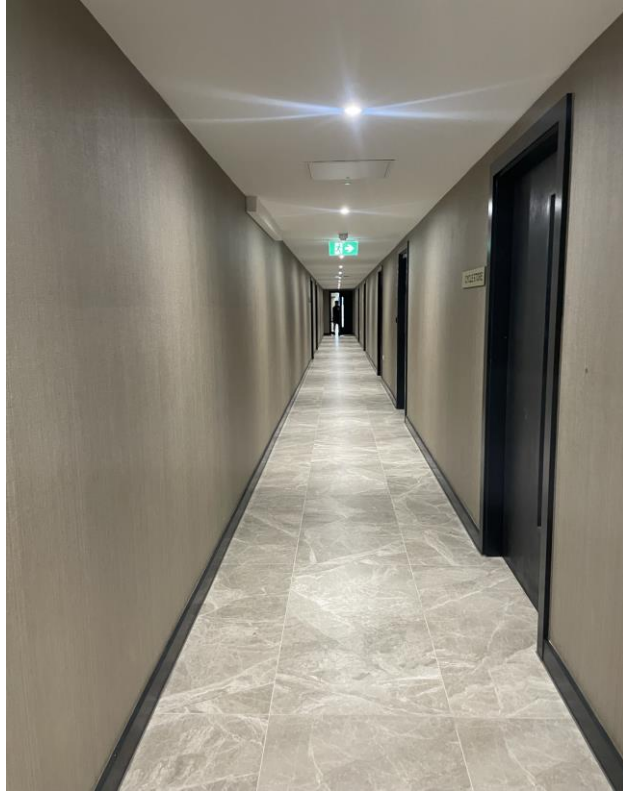
Ground Floor – Corridor finishes
