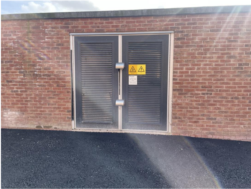
Sub-station louvre doors installed
