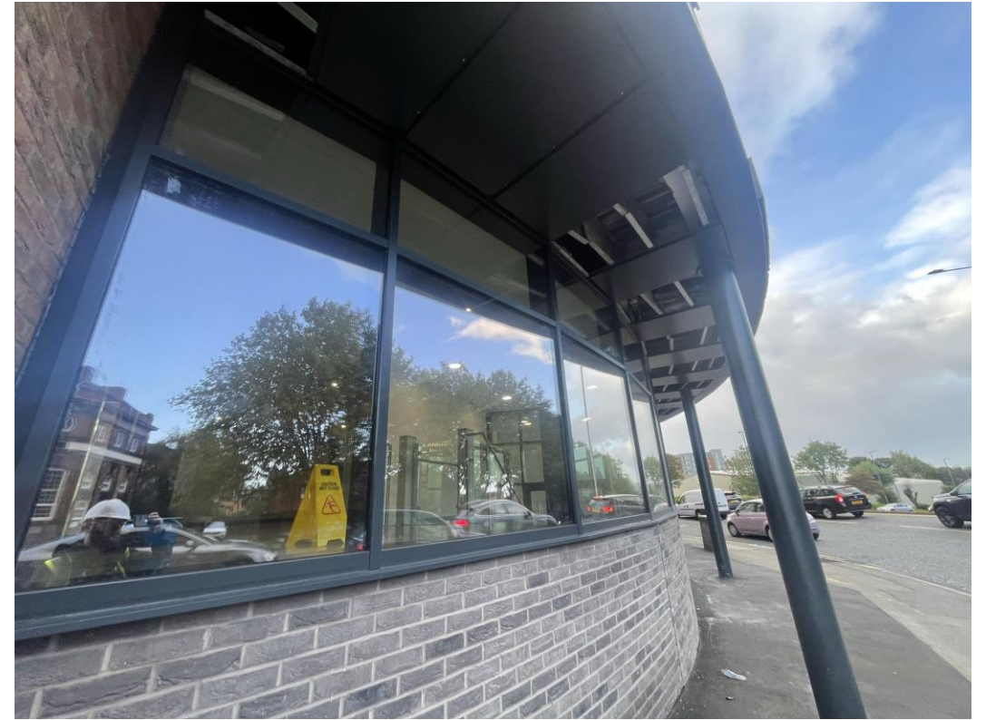
Main Entrance – Curtain Walling
