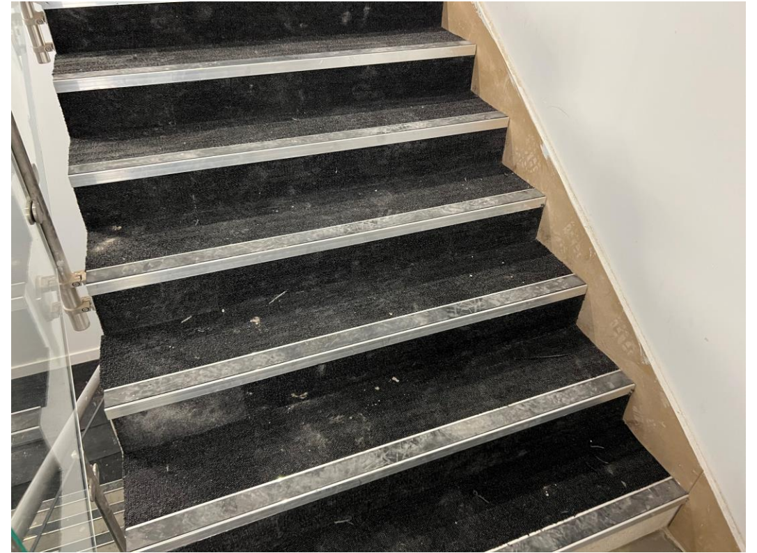
Stair Core – Carpet finishes installed
