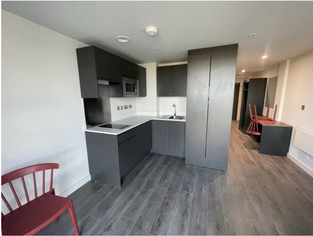
Residential Block – Kitchen installation
