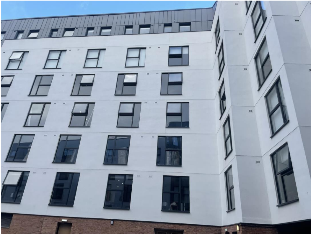
Residential Block – Infill of hoist apartments complete
