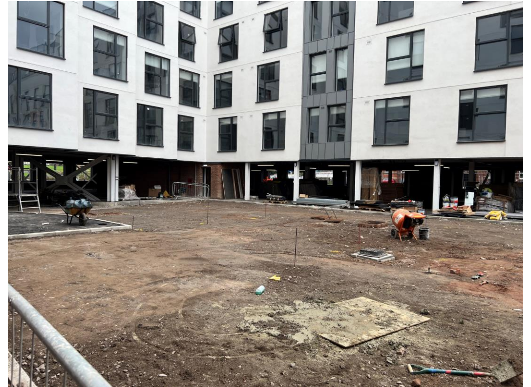
Preparation works for tarmac road surface
