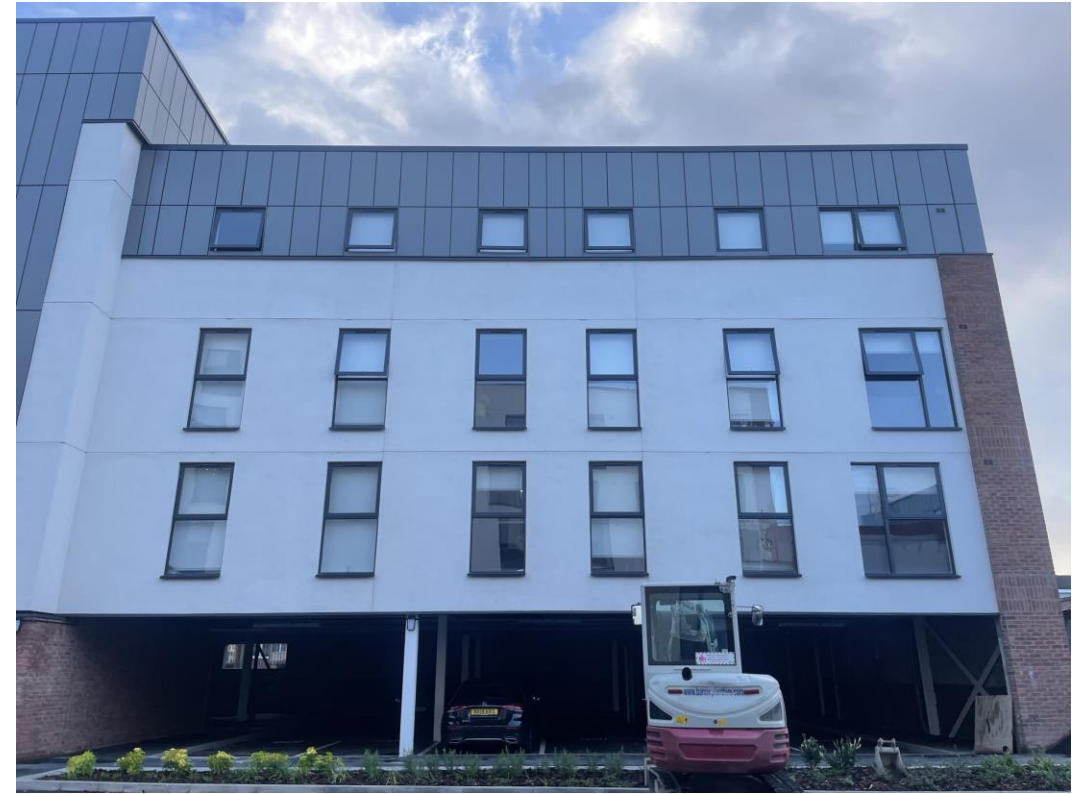
Student Block – External façade complete
