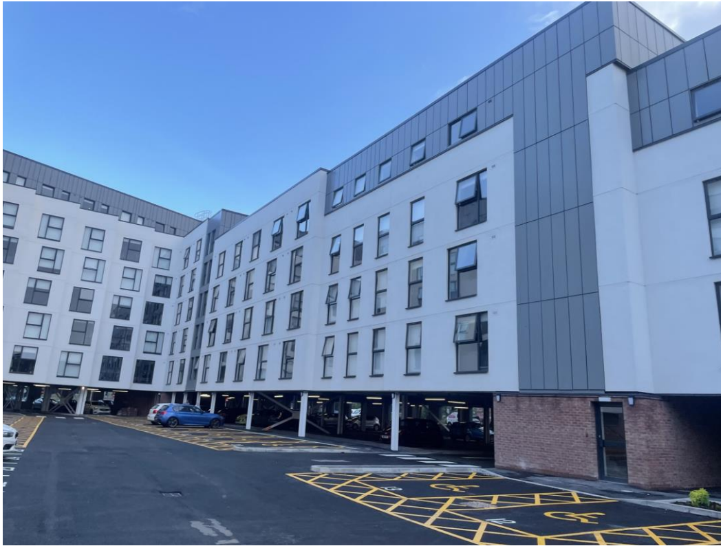
Student Block – External façade complete
