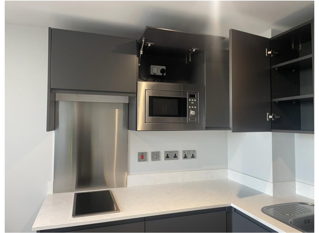
Residential Block – Kitchen installation
