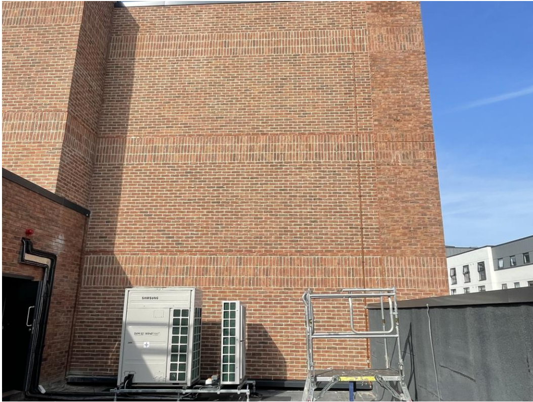
Residential - Brick slip installation complete
