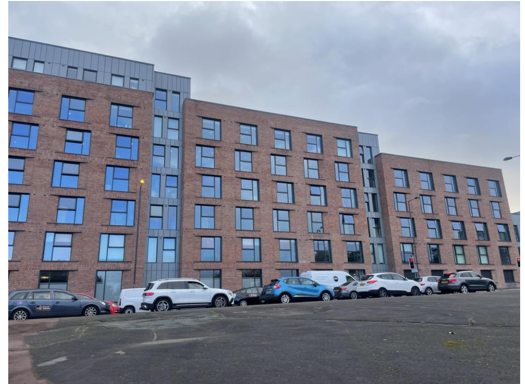
Brunswick Road – Rainscreen cladding
