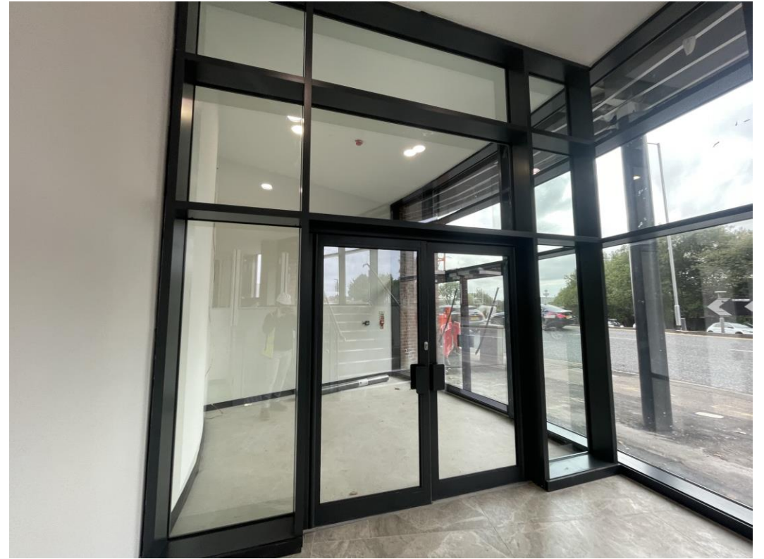
Maine Entrance – Curtain walling
