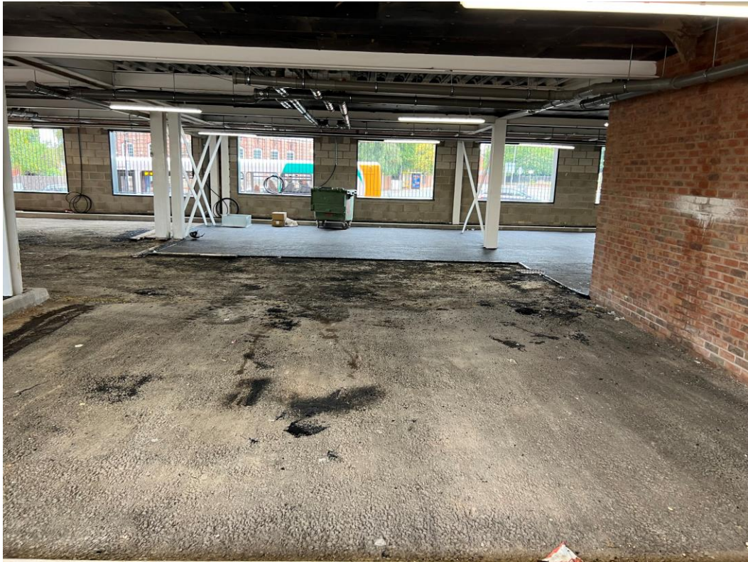
Basecoat tarmac for road surface
