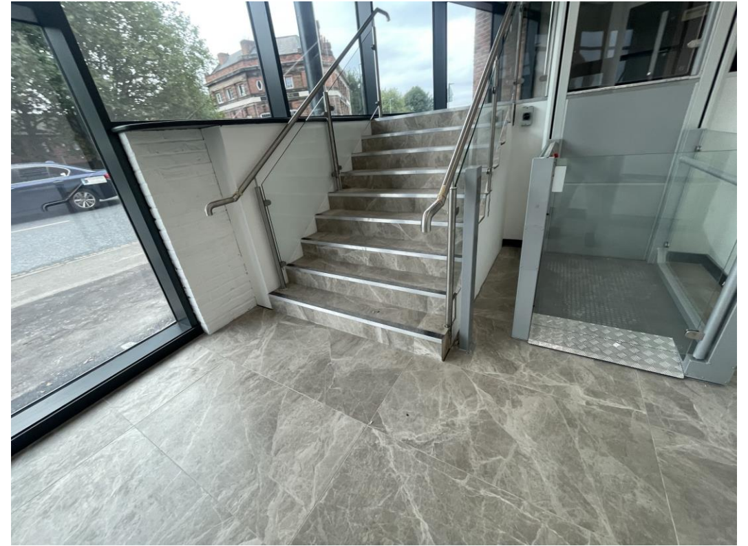
Maine Entrance – Staircase finishes
