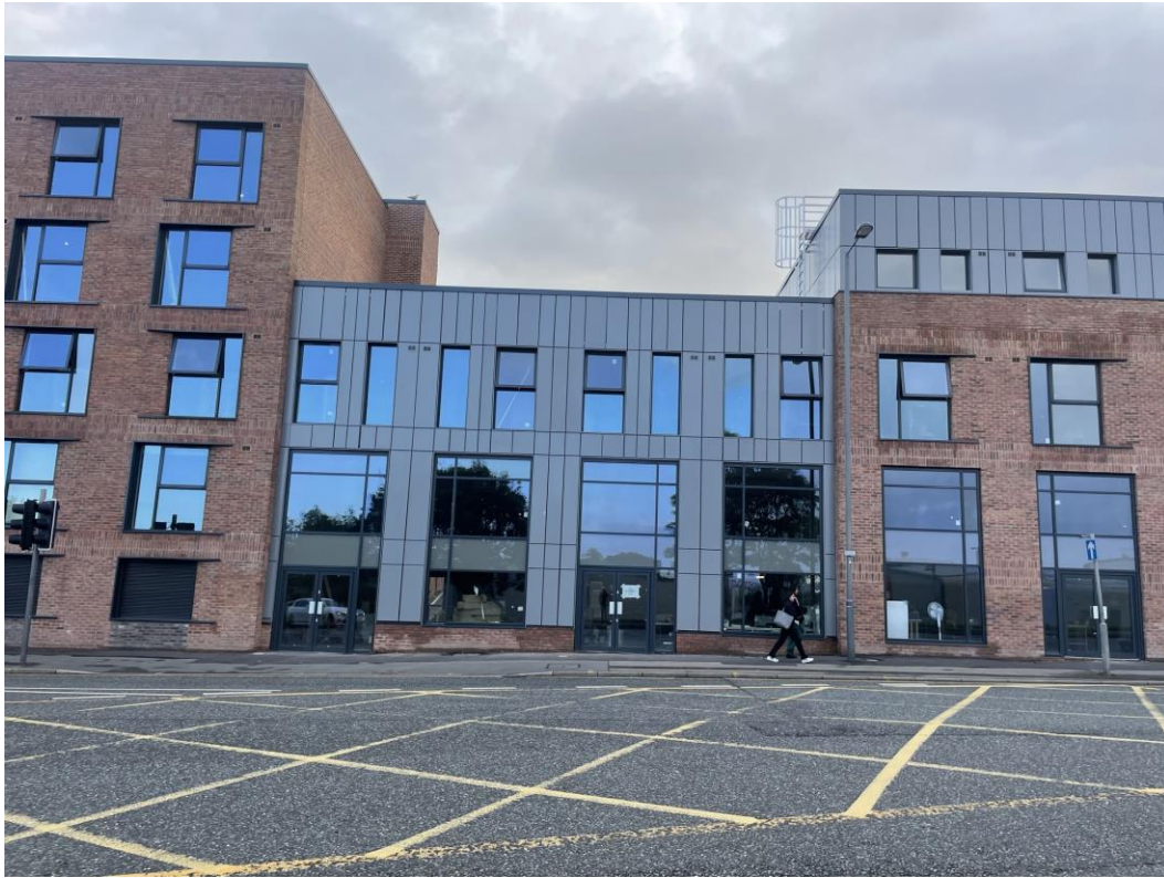
Commercial Block - Curtain walling
