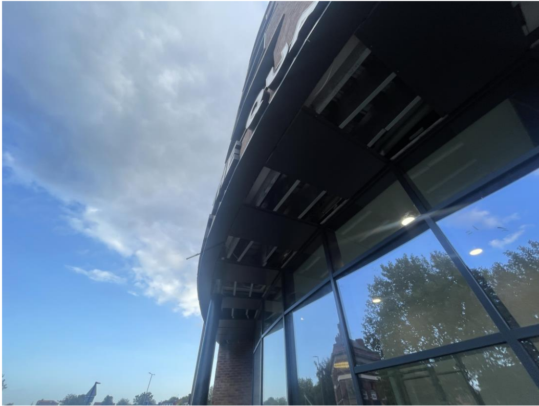
Main Entrance – Soffit detail nearing completion
