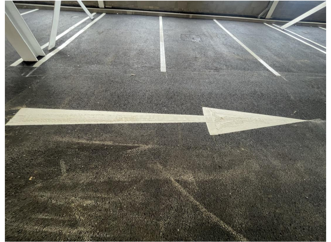
Vehicle directional markings in place
