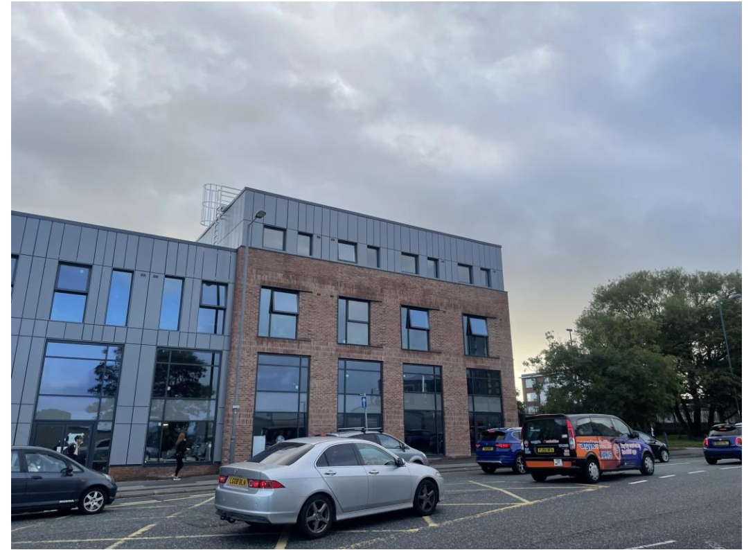
Commercial Block - Curtain walling
