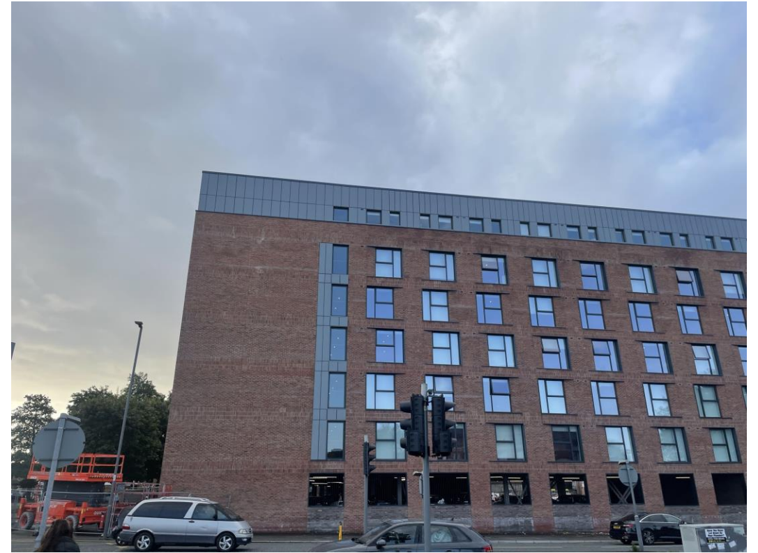
West Derby Road - Site view
