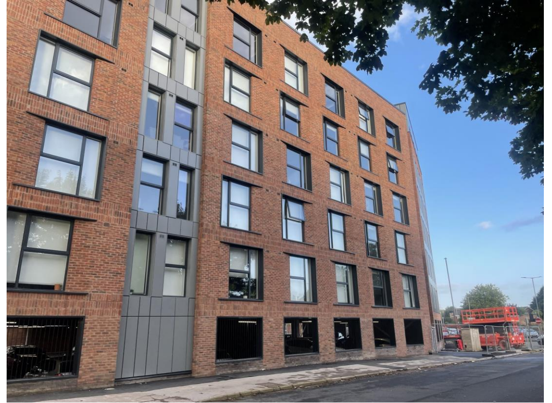
Walker Street - Site view
