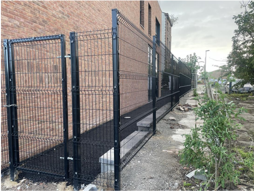
Metal fencing in place
