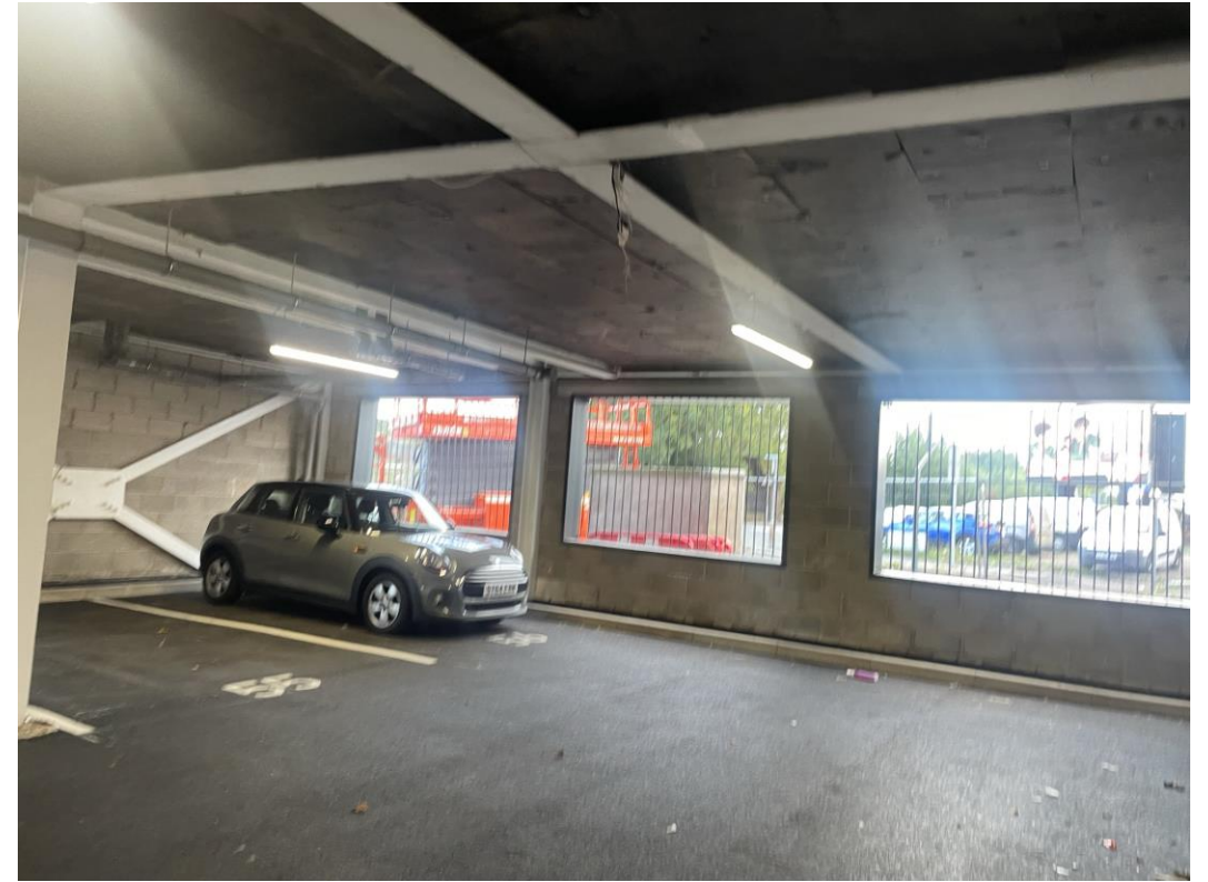
Ceiling soffit insulation detail installed
