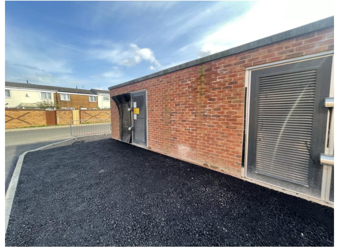
Sub-station louvre doors installed
