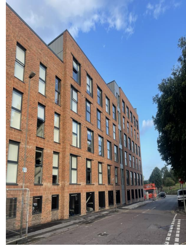
Walker Street - Site view
