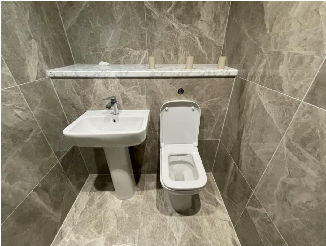
Ground Floor WC – Sanitary Items
