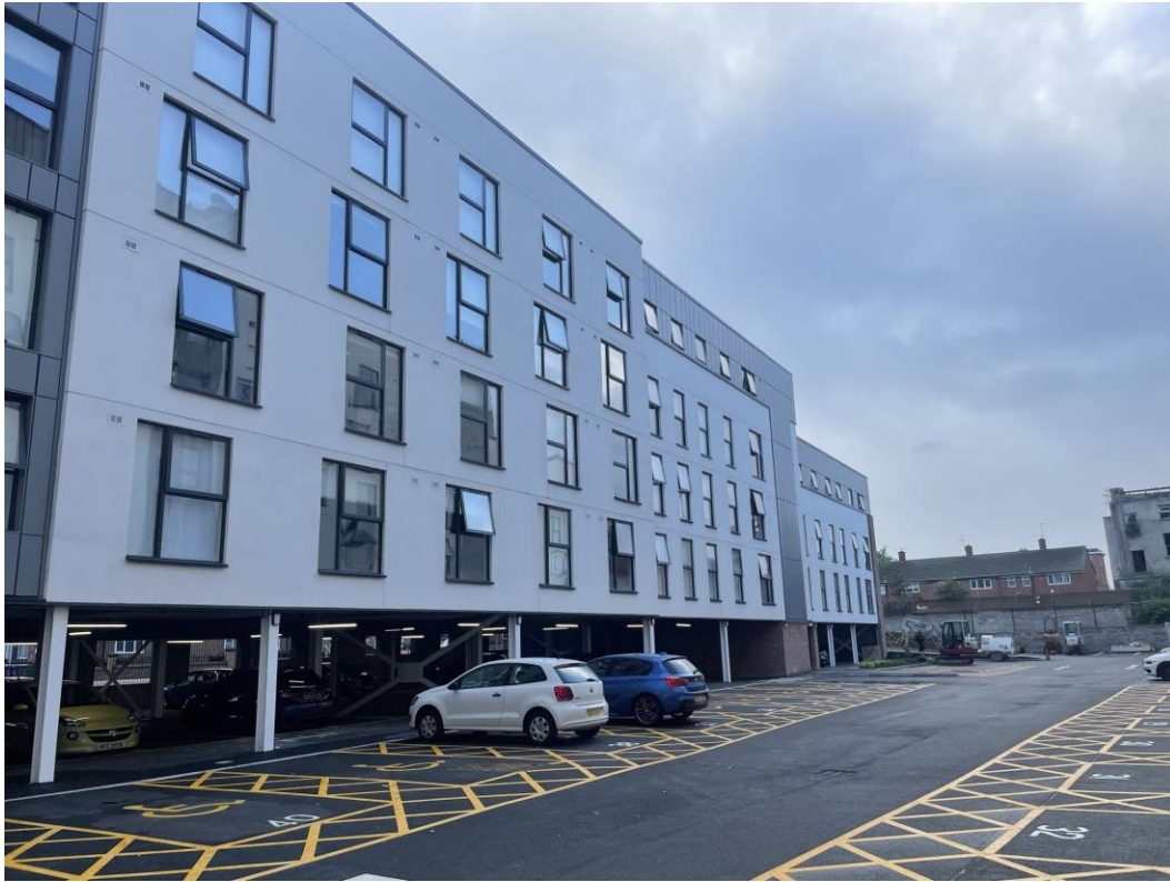
Student Block – External façade complete
