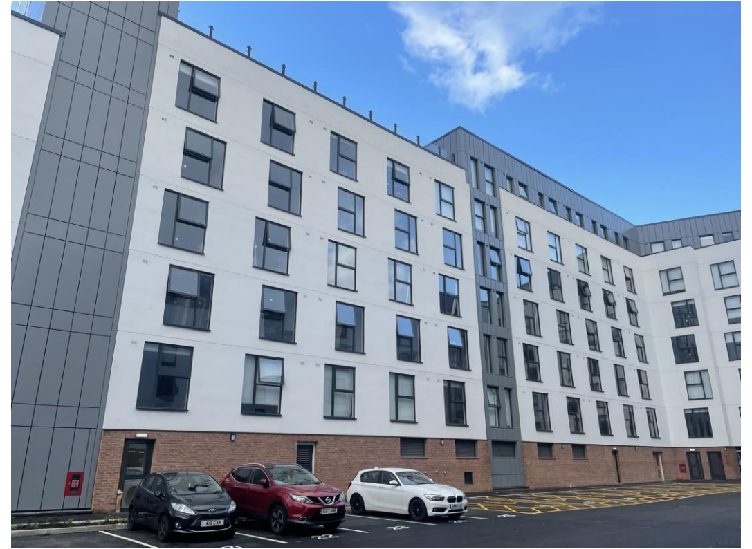
Residential Block – External façade complete
