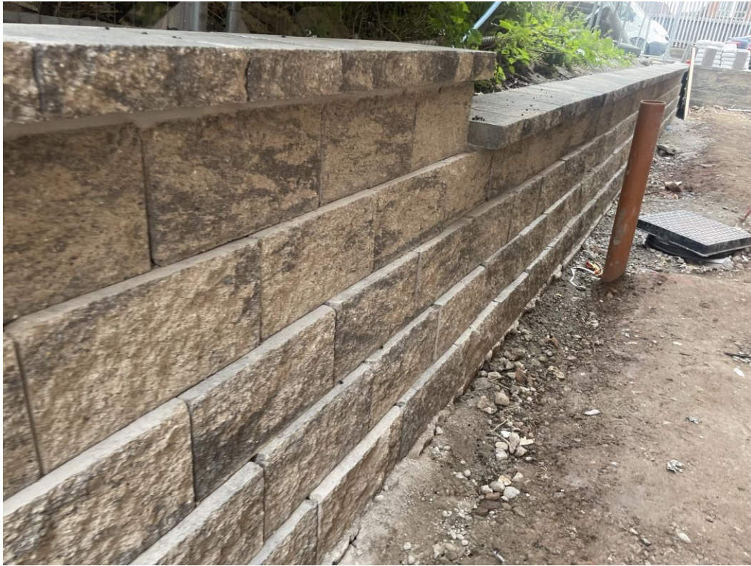
Retaining wall complete
