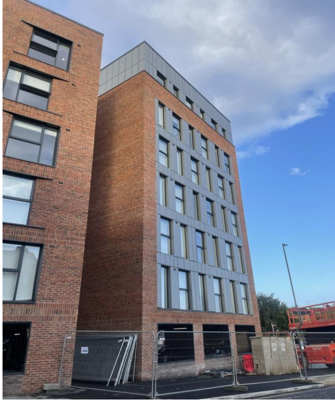
Walker Street - Site view
