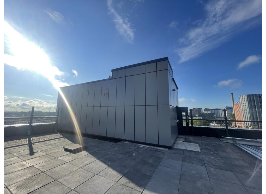
Residential Block – Rainscreen cladding
