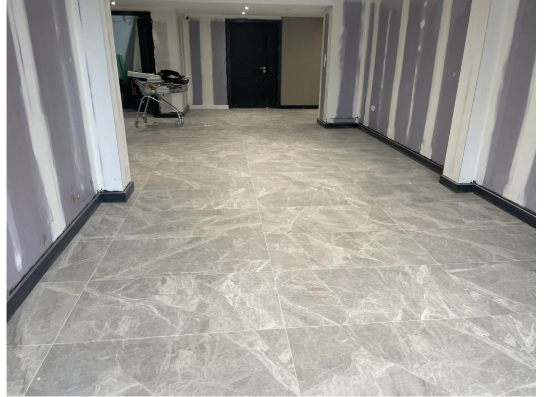
Ground Floor – Floor tiling installed
