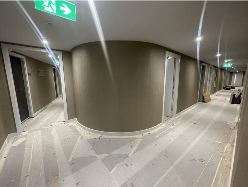
Student Block – Corridor wallpaper applied
