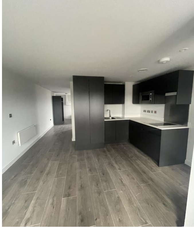
Residential Block – Decoration works on-going
