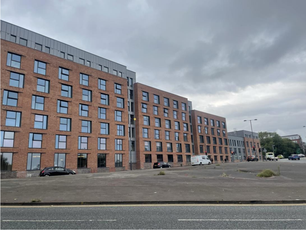
Brunswick Road – Site view
