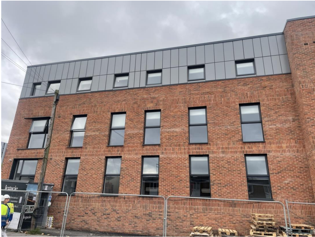
Walker Street - Site view
