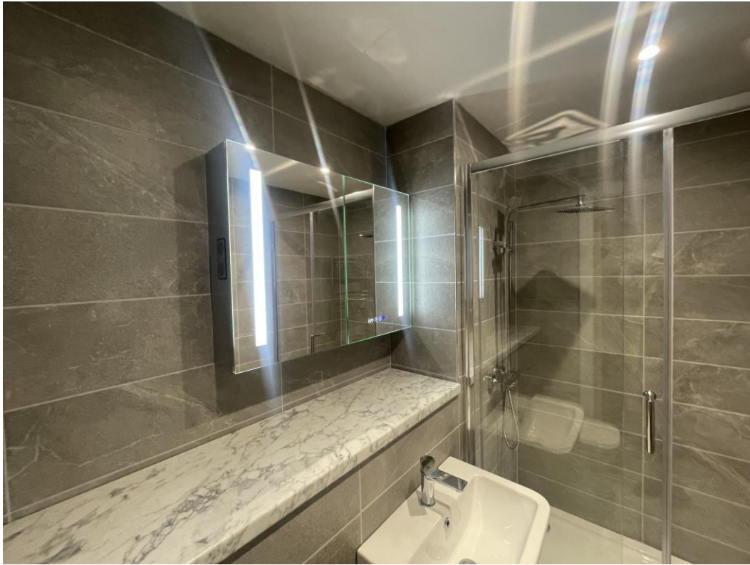
Residential Block – Mirror installed
