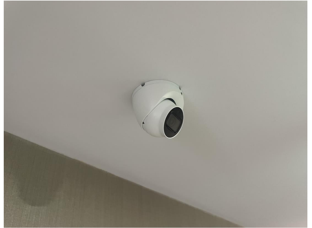
Residential Block – CCTV
