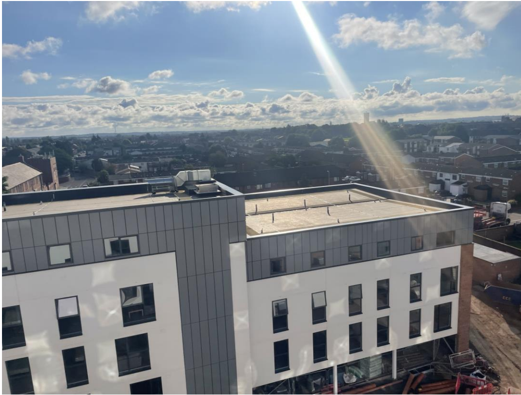
Student Zone – Rainscreen cladding complete
