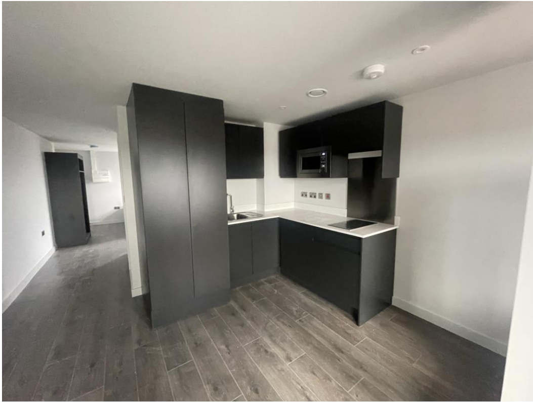
Residential Block – Kitchen installation
