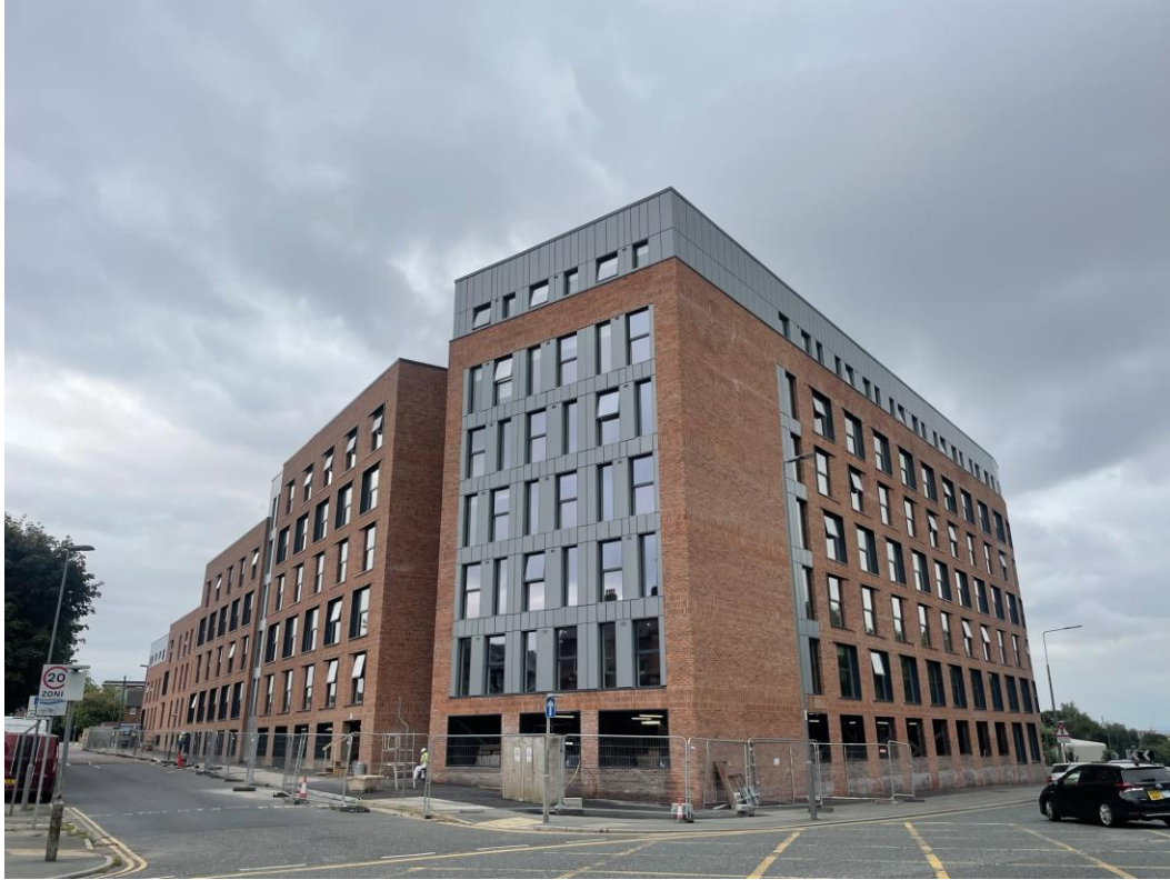
West Derby Road - Site view
