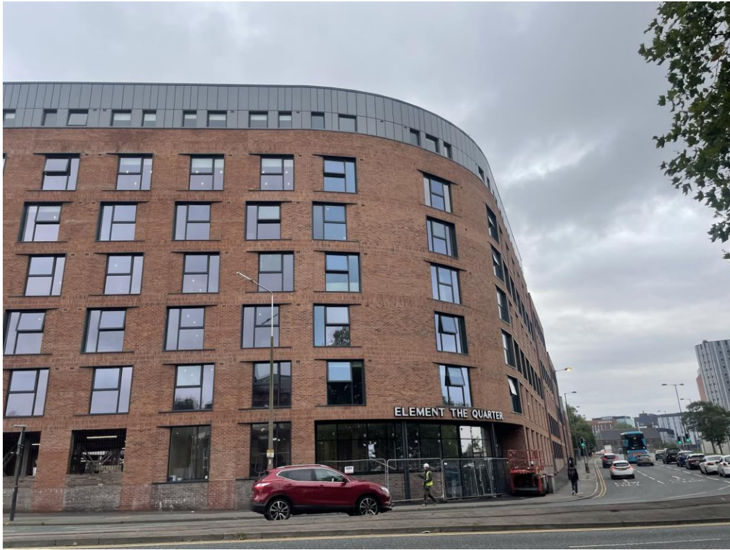
Brunswick Road – Building signage complete
