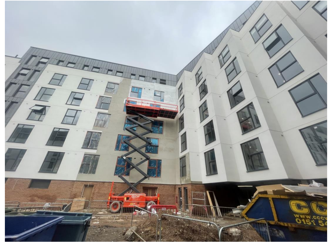
Residential Block – Application of topcoat of render on-going.
