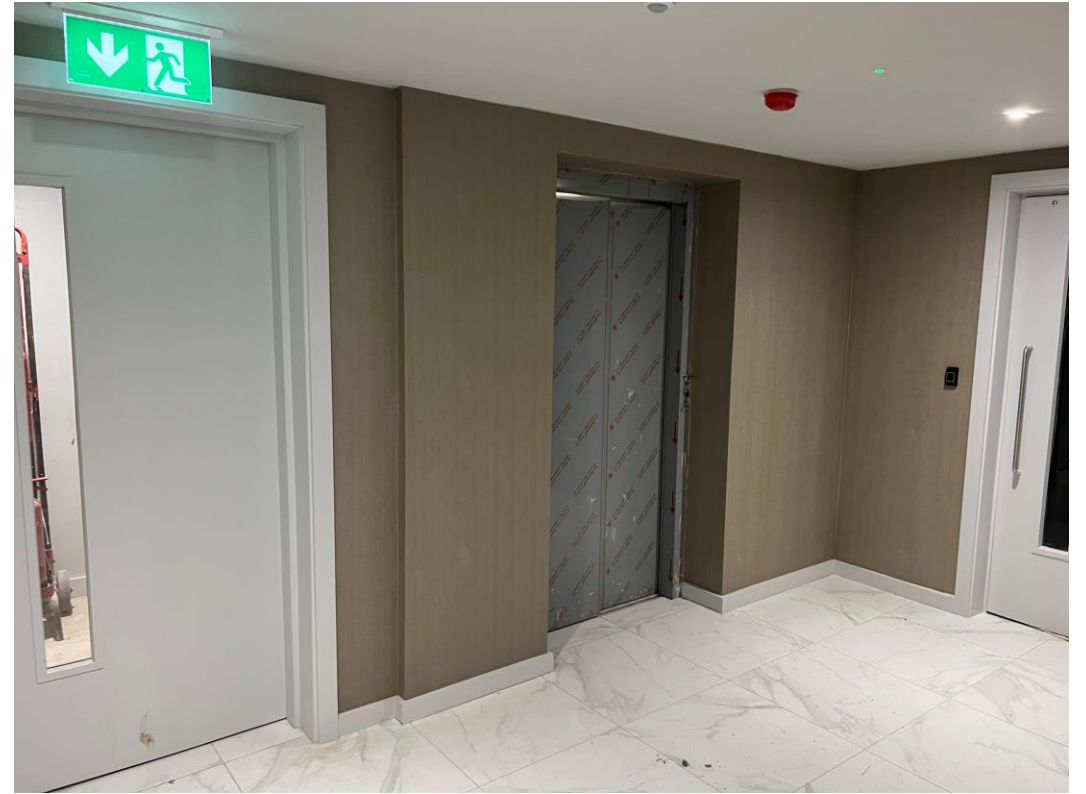
Residential Block – Lift lobby wallpaper
