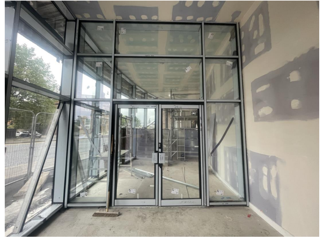
Ground Floor– Curtain walling installed
