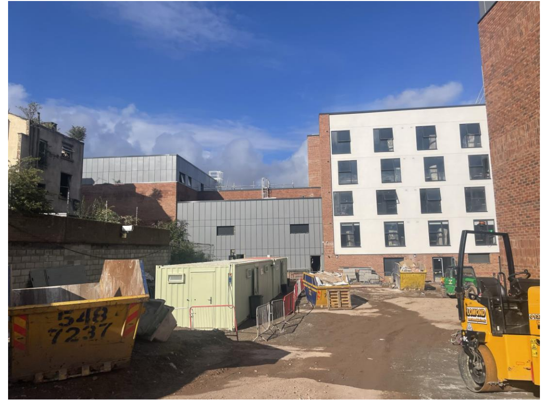
Commercial Zone – Rainscreen cladding complete
