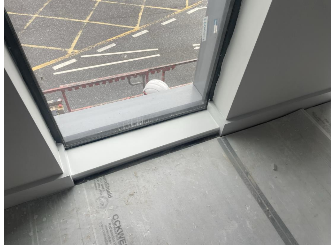
Residential Block – Window board installed & decorated
