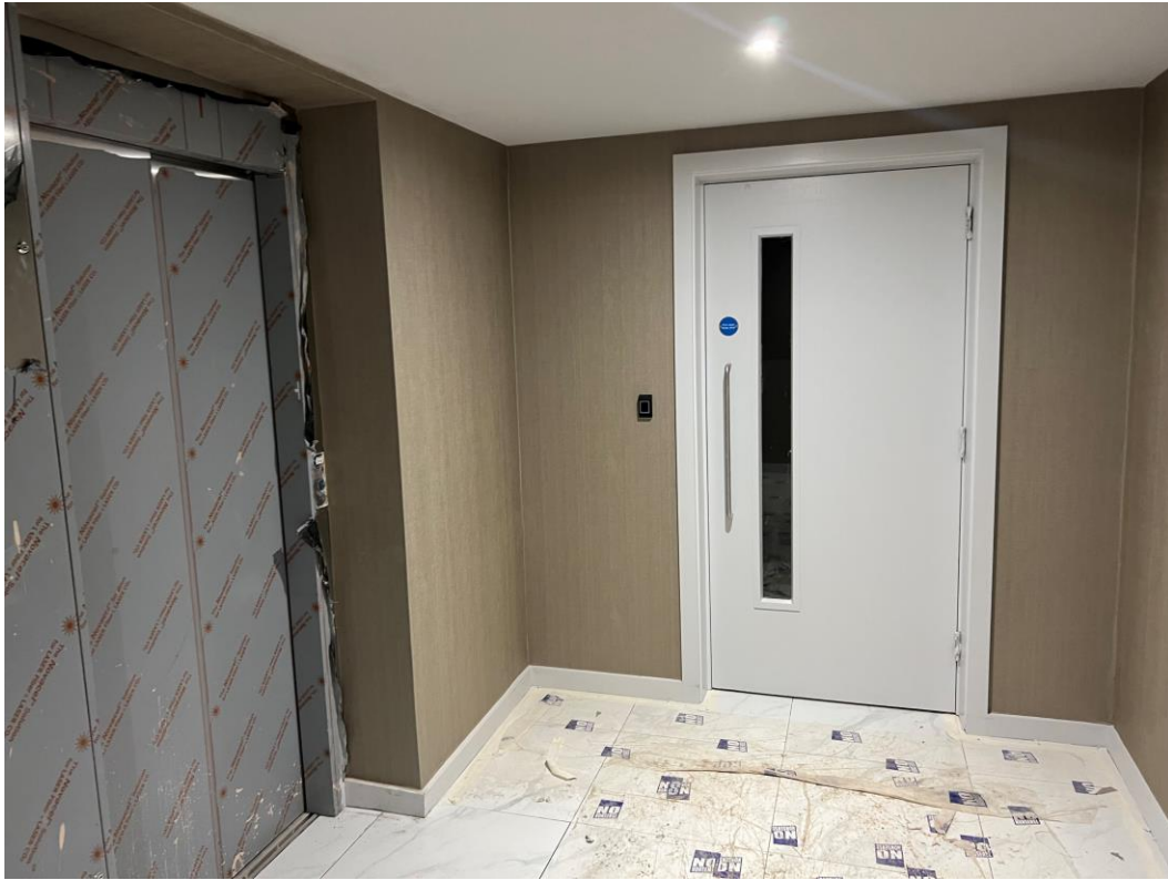
Residential Block – Lift lobby finishes
