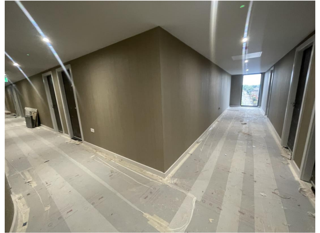
Student Block – Corridor wallpaper applied
