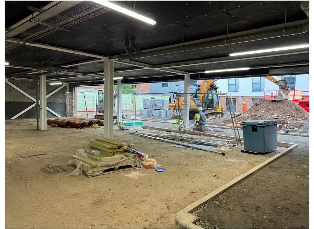
Ceiling soffit insulation detail installed
