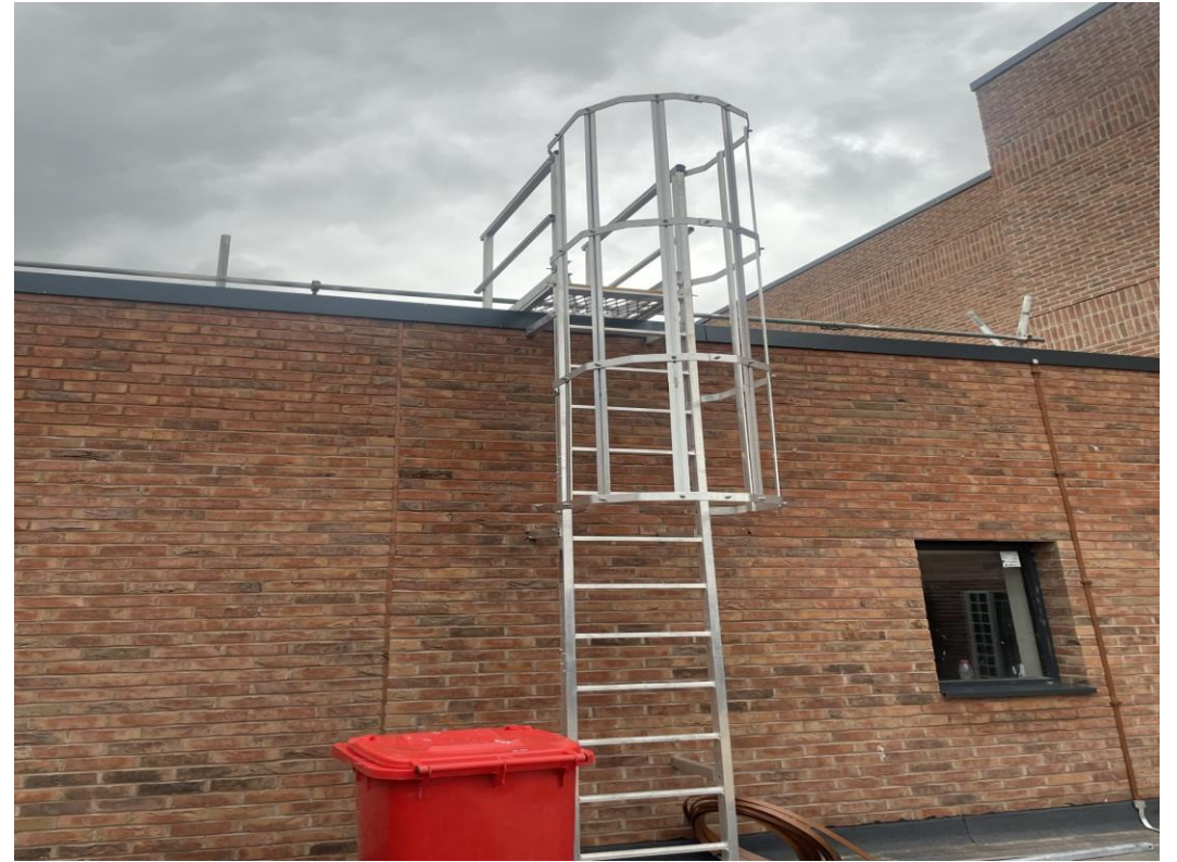
Fixed ladder access
