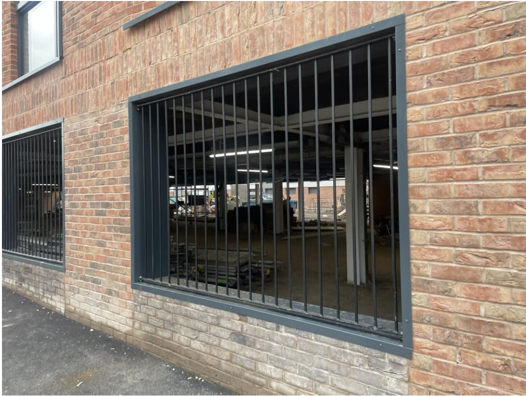
Undercroft parking – Railings & reveal trim
