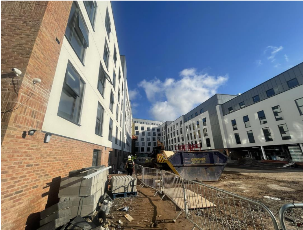
Viewed from site compound
