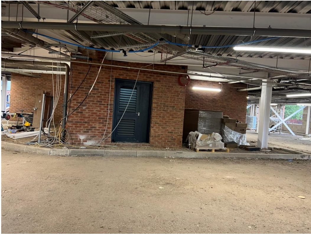
Undercroft Parking – Site view
