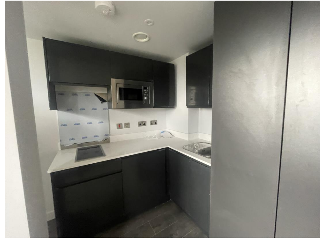
Residential Block – Kitchen installation
