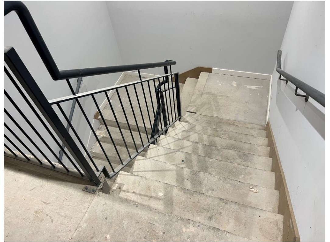
Residential Block – Handrails & balustrades
