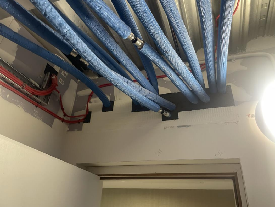
Residential Wing – Fire Stopping
