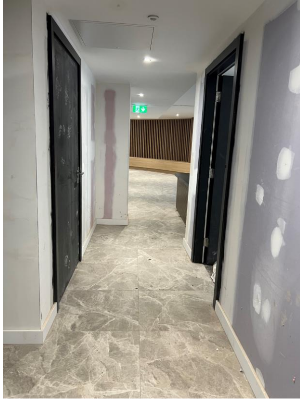
Ground Floor – Floor tiling installed
