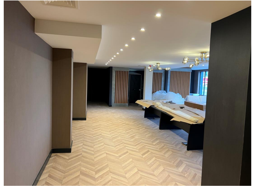
Ground Floor Study – Furniture installation commenced
