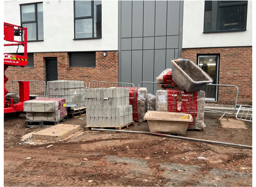
Materials Stored – Concrete kerbs
