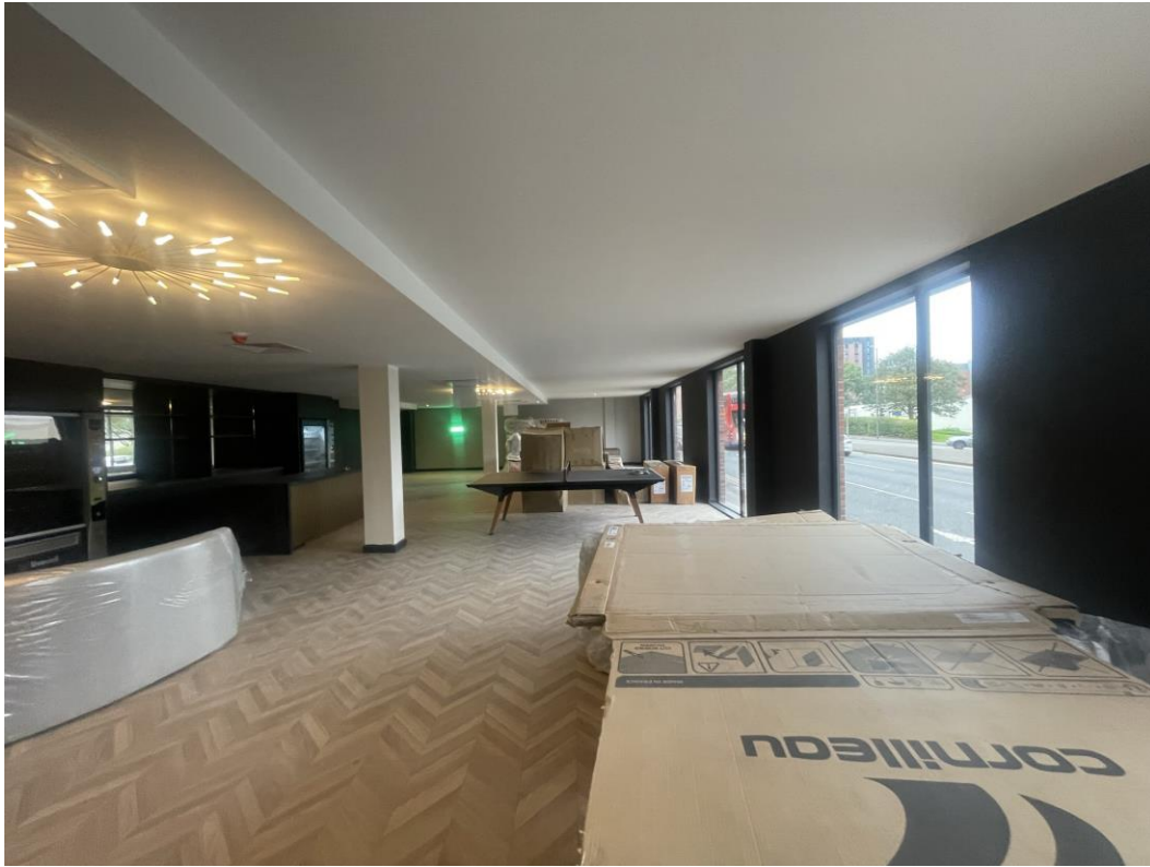
Ground Floor Games / Lounge – Furniture installation commenced
