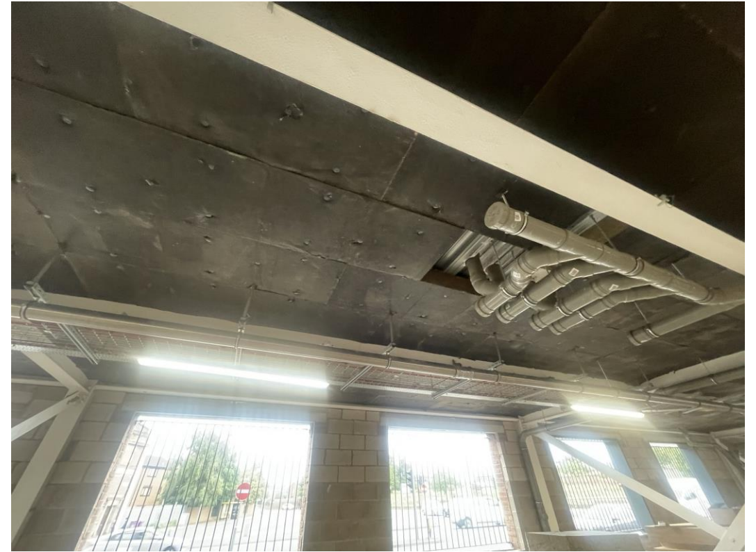
Ceiling soffit insulation detail installed
