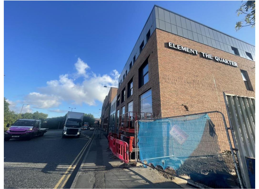
Commercial Block - Curtain walling
