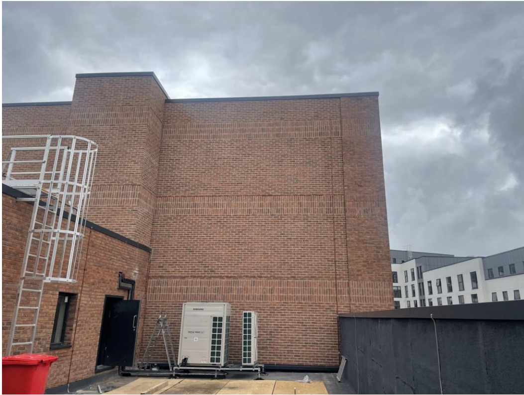
Residential - Brick slip installation complete
