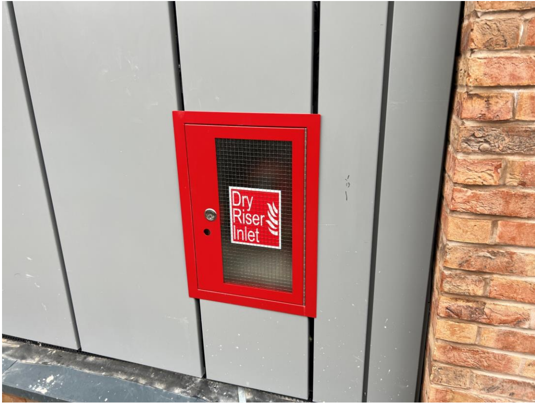
Dry riser installation complete
