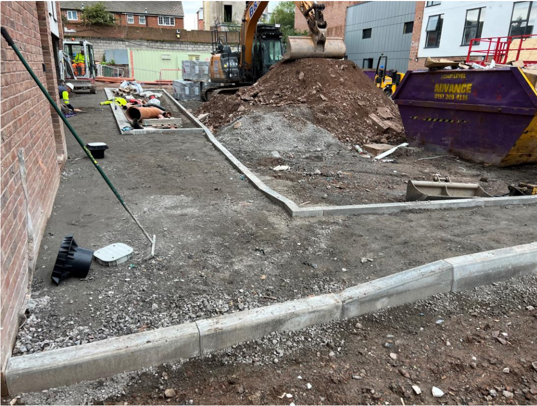
Kerb line installation and surface preparations works on-going
