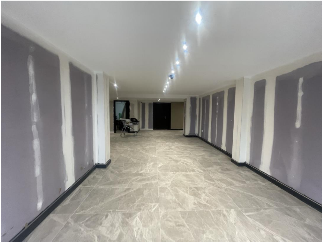
Ground Floor – Tape & jointing to Corridor walls & ceilings
