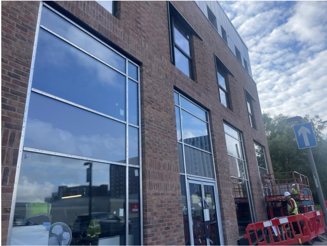
Commercial Block - Curtain walling
