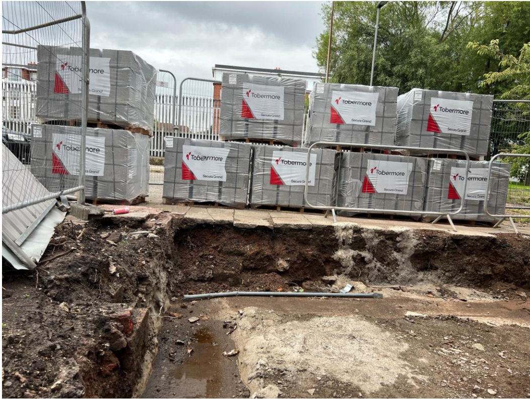
Material storage – Concrete blocks
