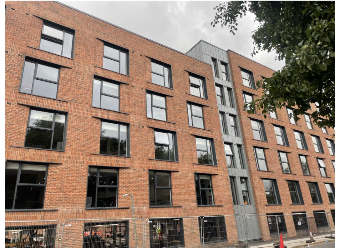
Walker Street - Site view
