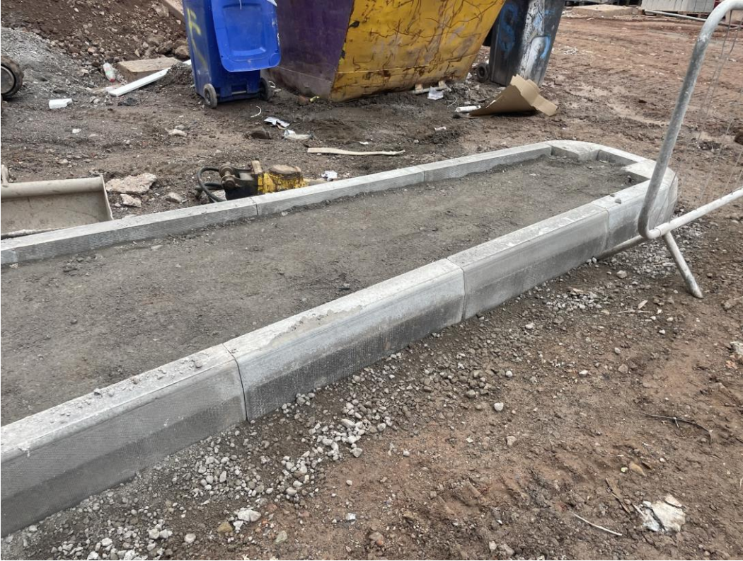
Kerb line installation on-going
