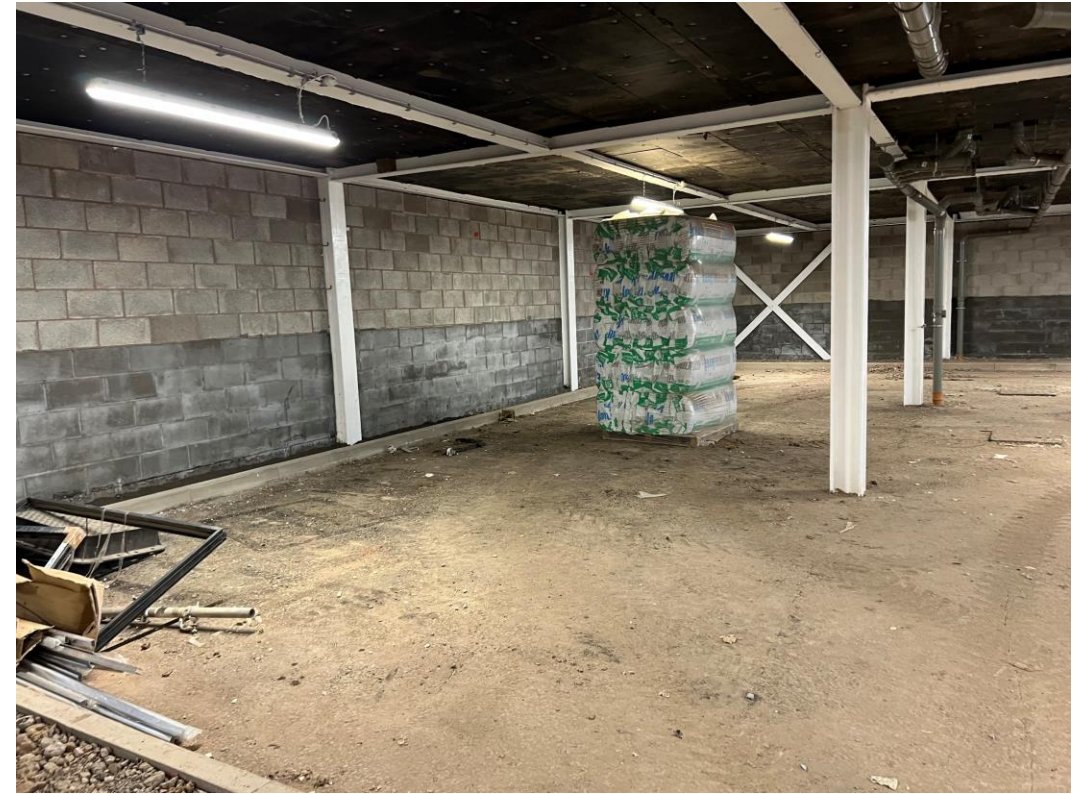
Tanking slurry applied to blockwork
