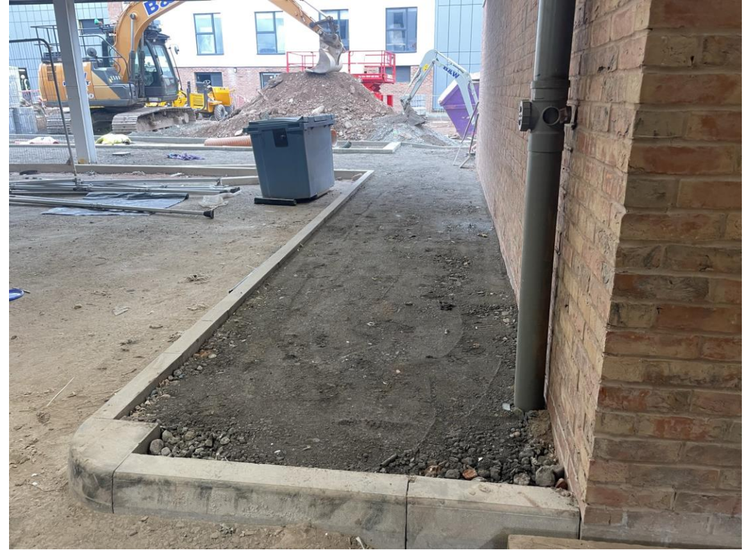
Base coat tarmac applied to newly formed footpaths
