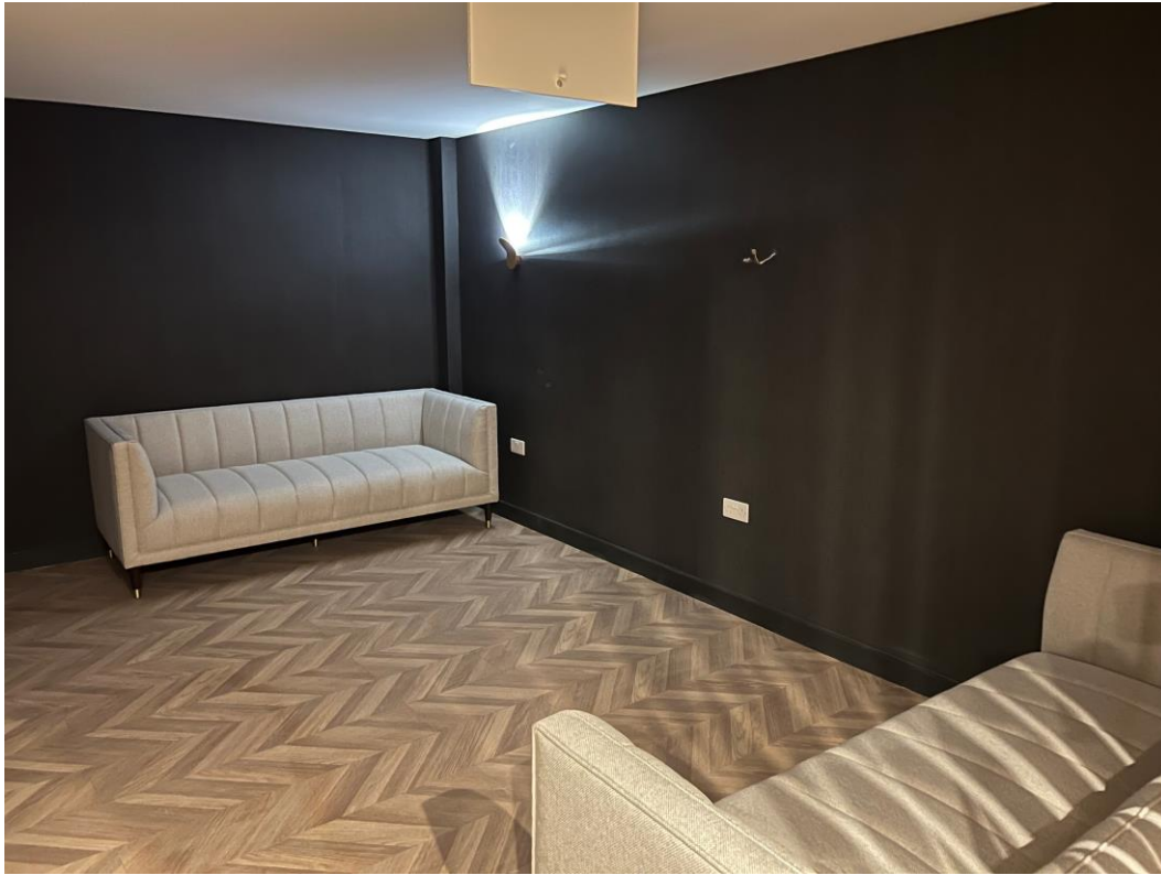
Ground Floor Study – Furniture installation commenced
