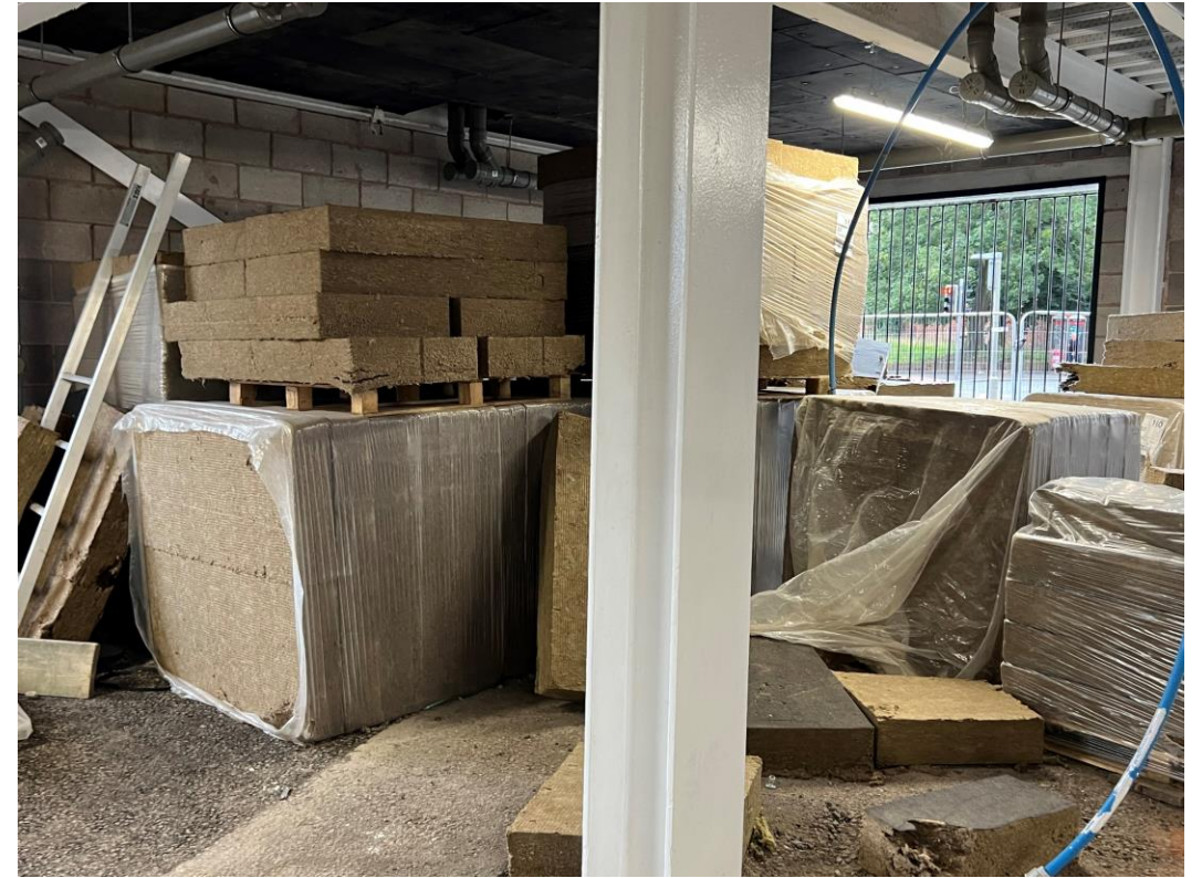
Material Storage – Soffit insulation
