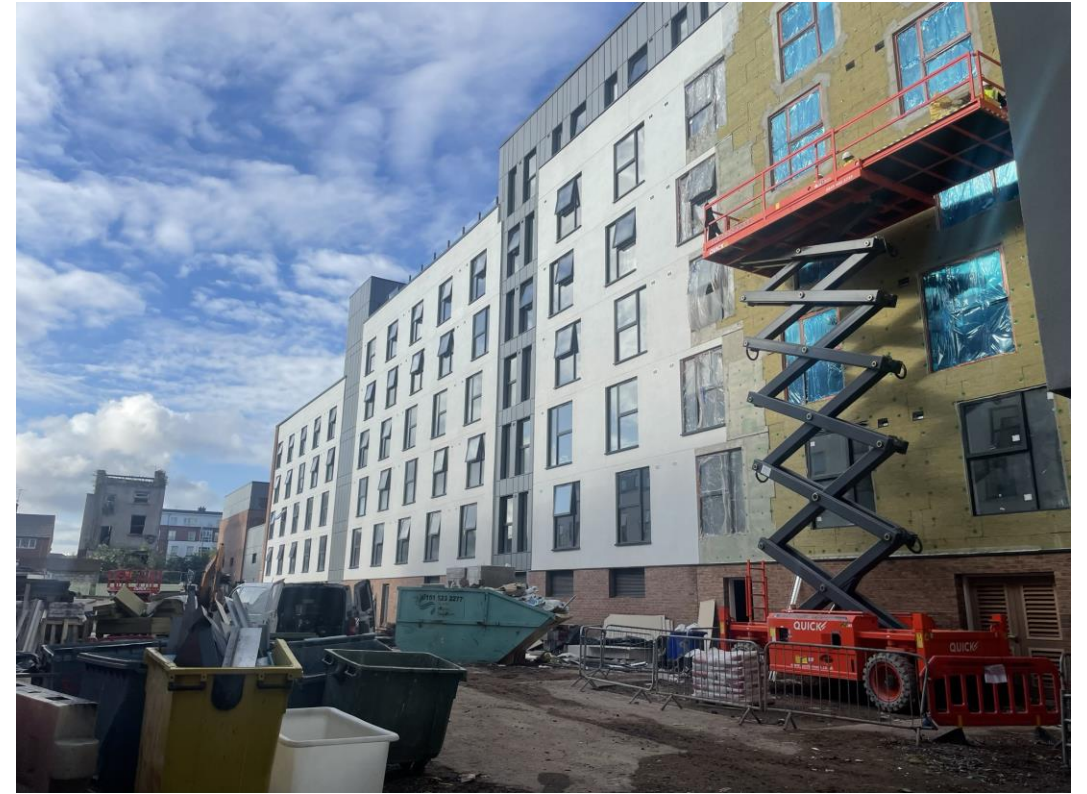
Residential Zone – Rainscreen cladding complete
