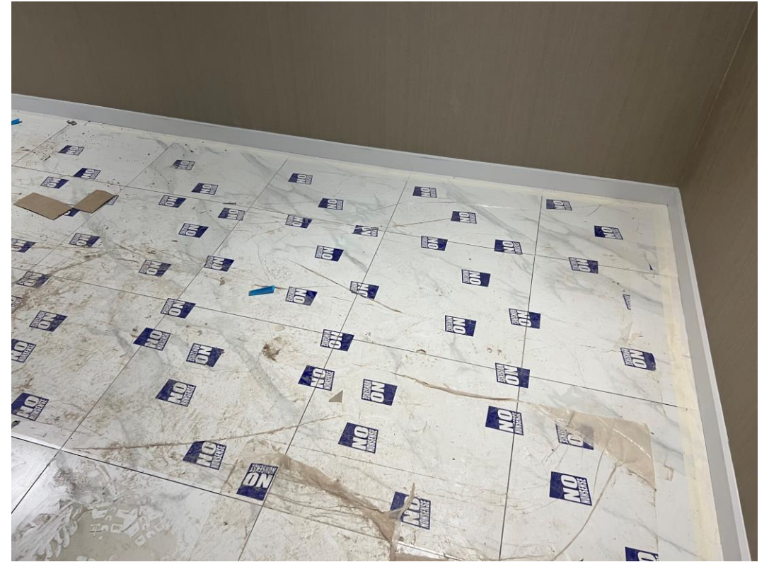
Residential Block – Lift lobby floor tiled flooring
