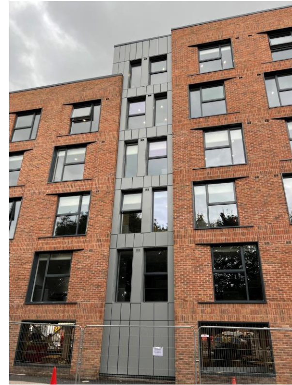
Brunswick Road – Rainscreen cladding
