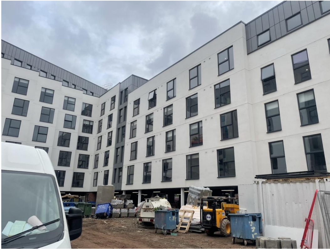
Student Wing – Cladding complete to internal courtyard
