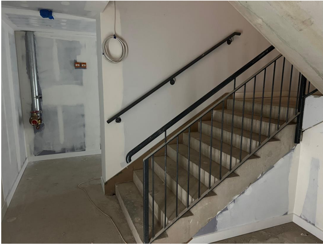
Student Block – Handrails & balustrades
