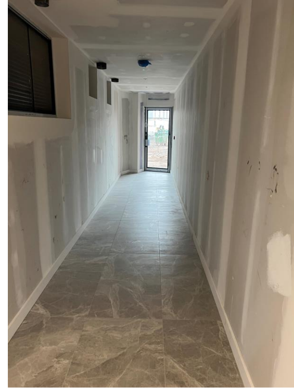
Ground Floor – Floor tiling installed
