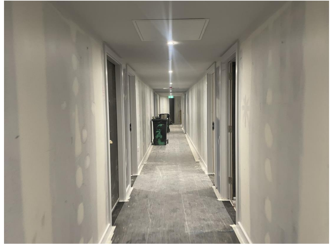
Ground Floor – Tape & jointing to Lobby walls
