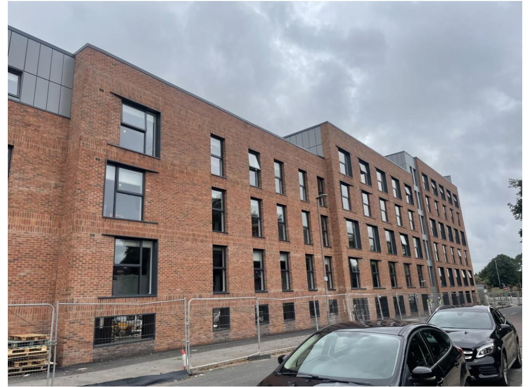
Walker Street - Site view
