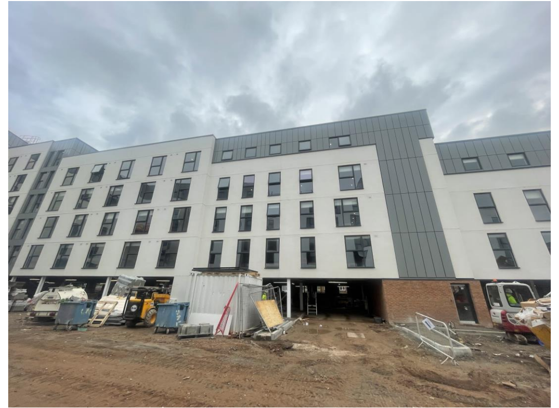
Student Wing – Cladding complete to internal courtyard
