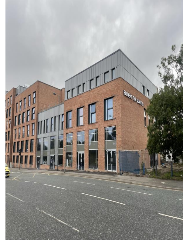
Curtain walling nearing completion
