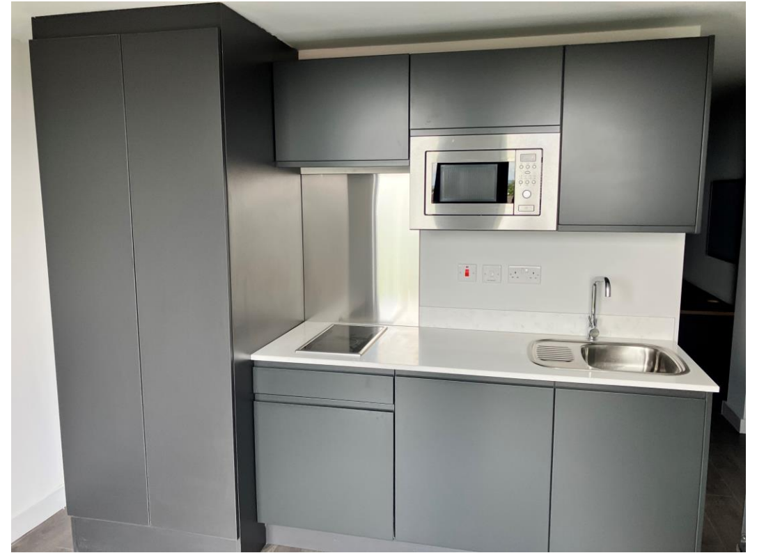
Residential Block – Kitchen installation
