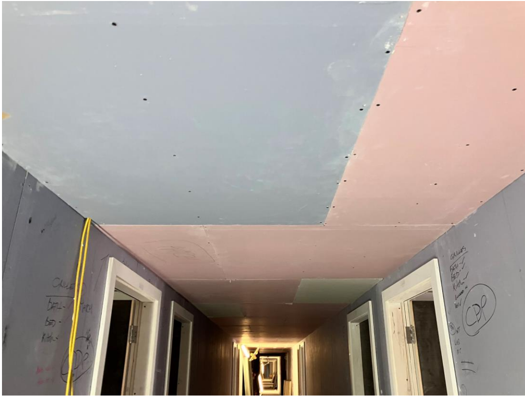
Residential Block – Corridor walls & ceilings boarded
