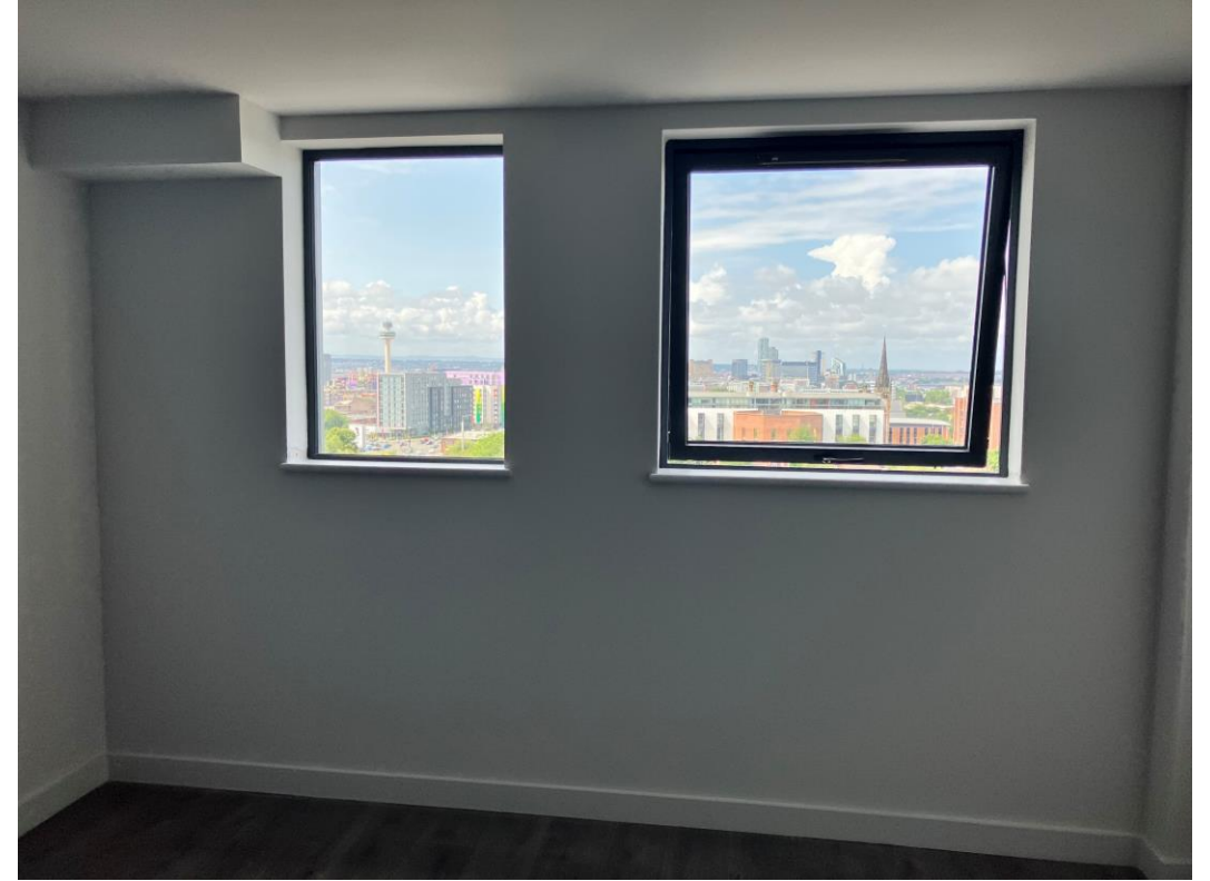
Residential Block – MDF Window boards
