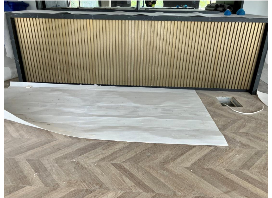
Ground Floor Games / Lounge – Kitchen area installation on-going
