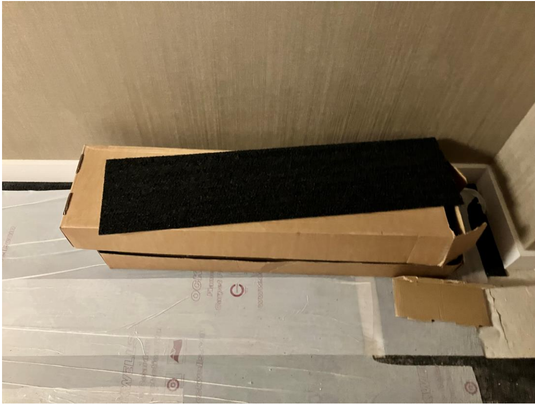
Material storage – Carpet Tiles
