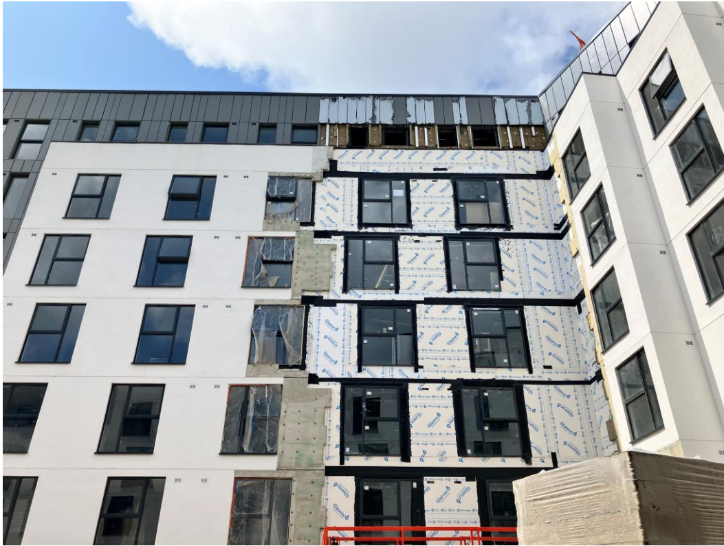
Residential Block – Infill of hoist apartment on-going
