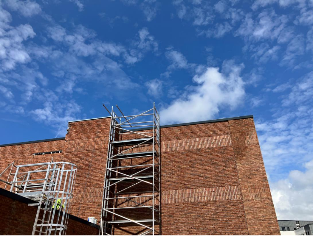
Residential - Brick slip installation on-going
