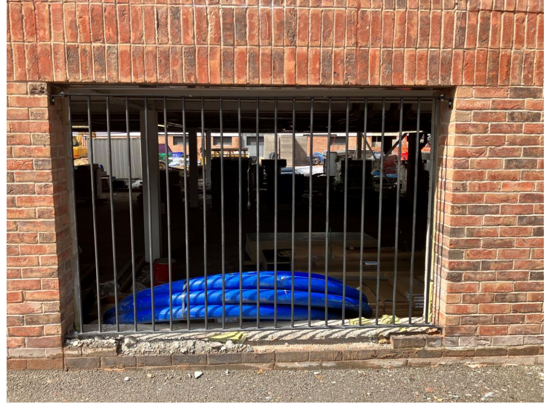
Undercroft parking - Railings
