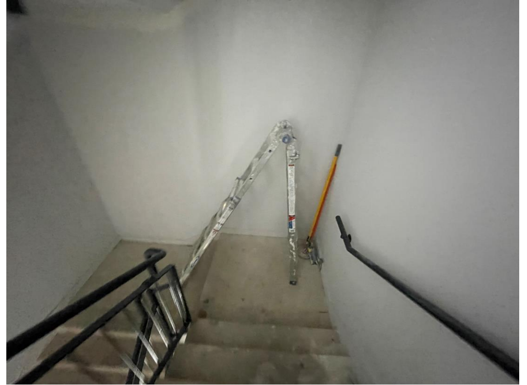
Residential Block – Decoration of stairwells on-going
