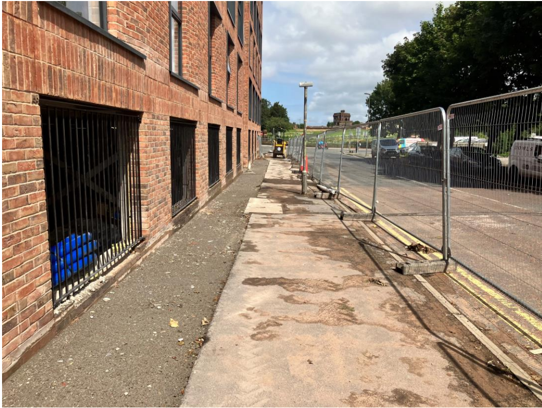
West Derby Road – Welfare & site cabins removed.
