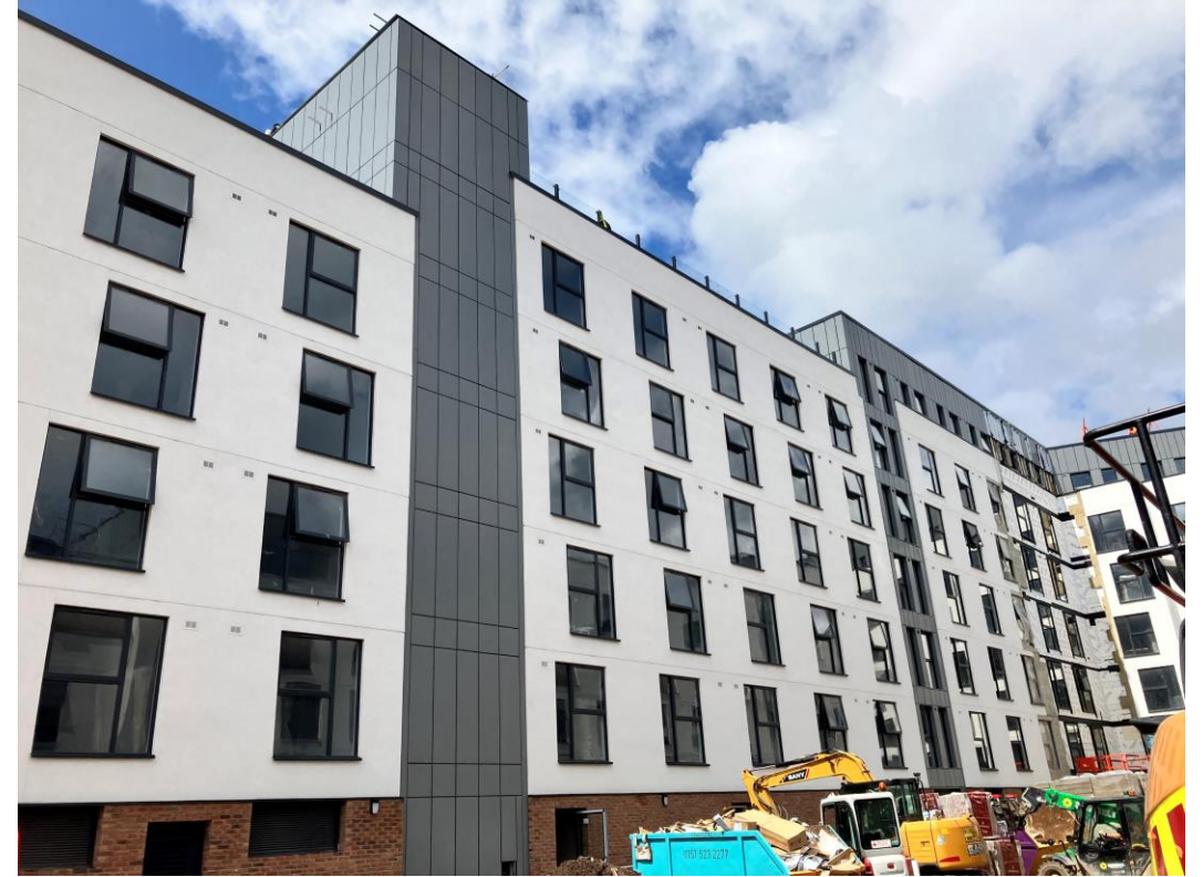
Residential Zone – Rainscreen cladding installation commenced
