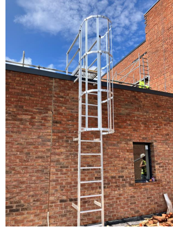
Fixed ladder access
