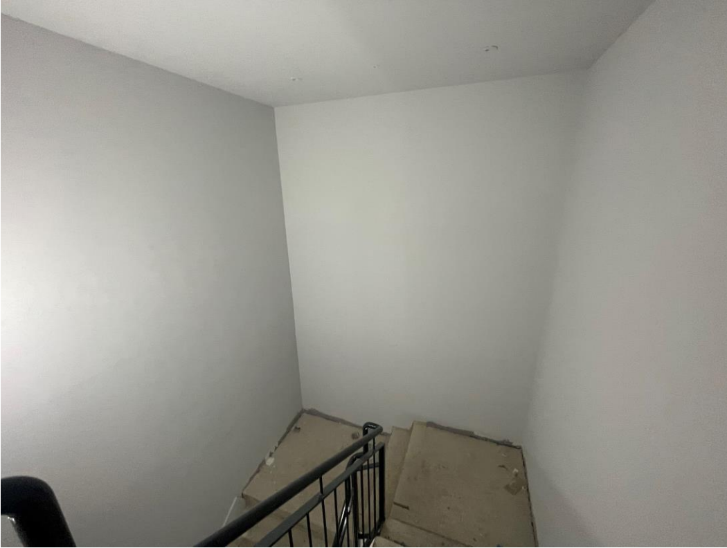
Residential Block – Decoration of stairwells on-going
