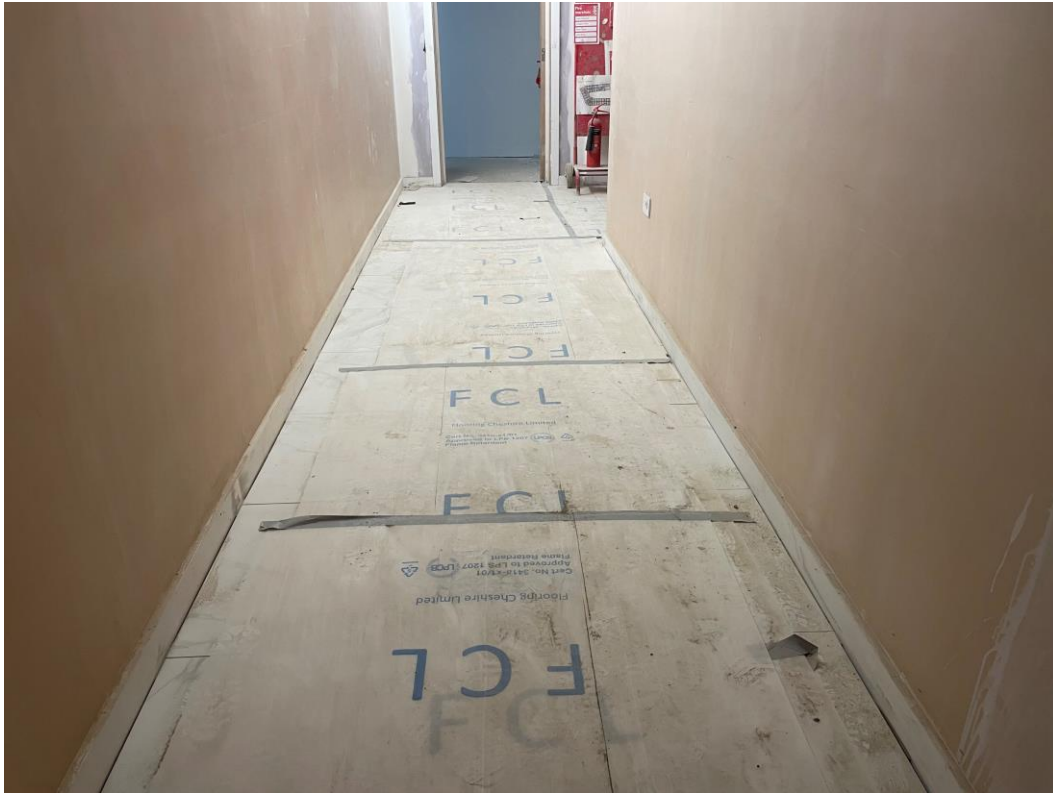
Residential Block – Lift lobby tiled flooring
