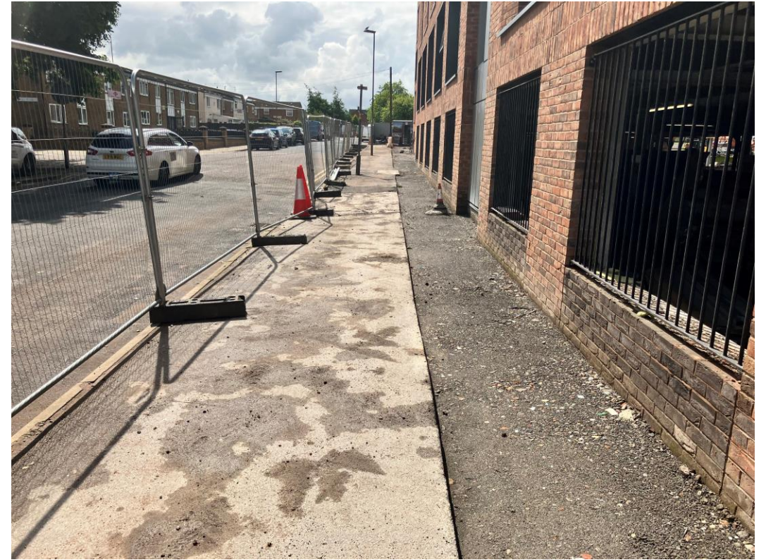
West Derby Road – Ground Works on-going
