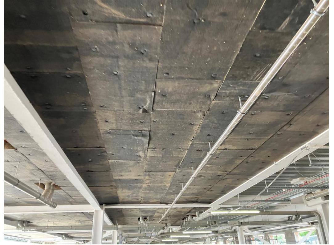
Ceiling soffit insulation detail installed
