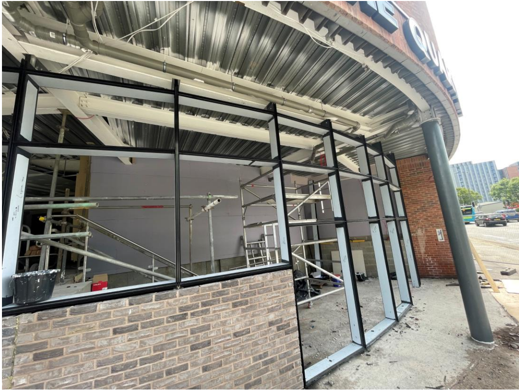
Main Entrance – Curtain wall installation
