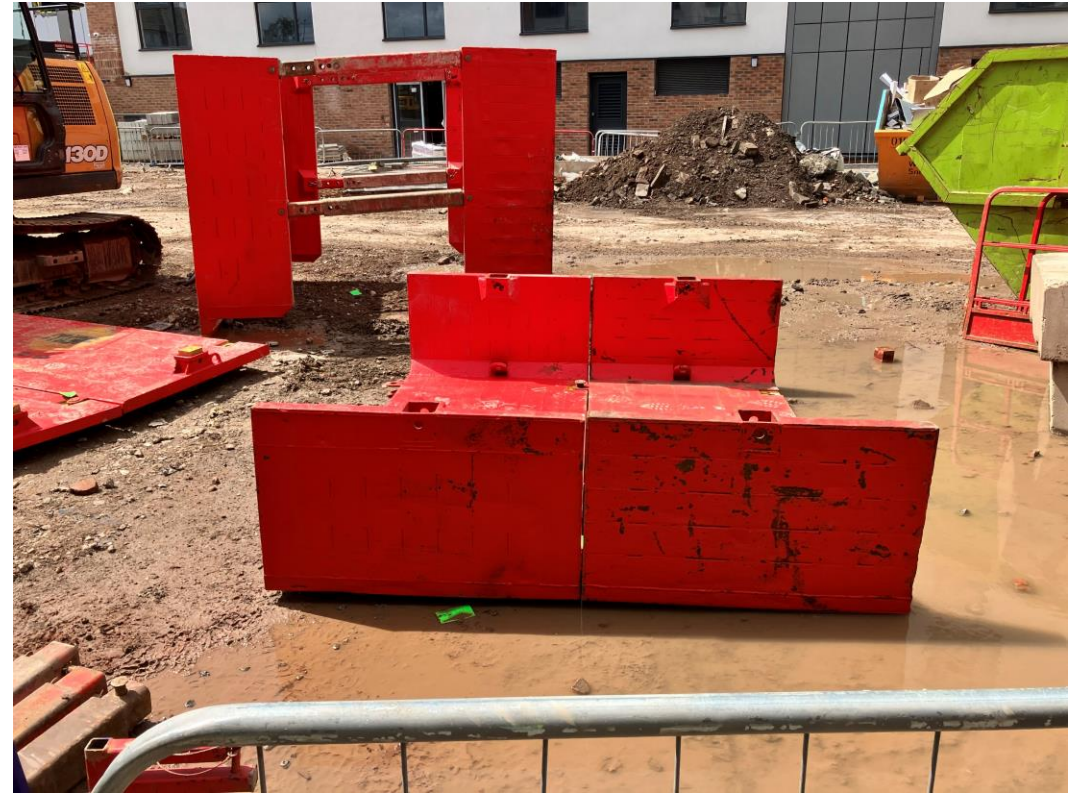
Excavation shoring boxes
