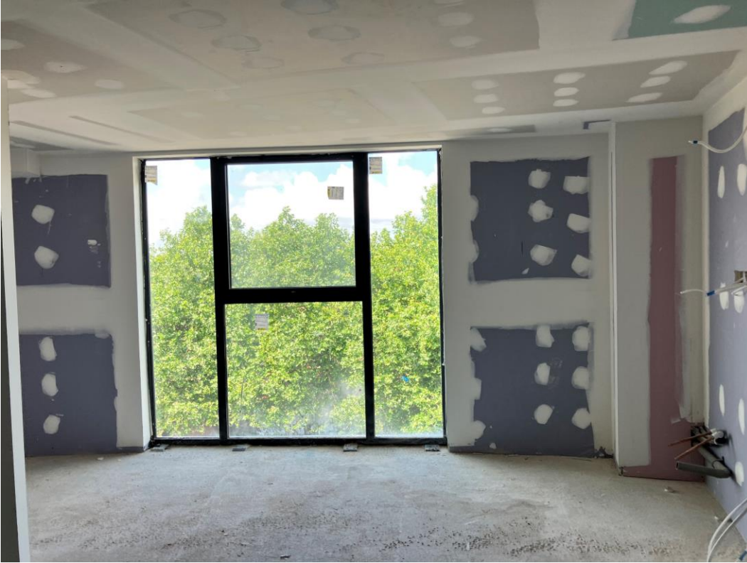
Residential Block – Walls & ceiling tape & jointed
