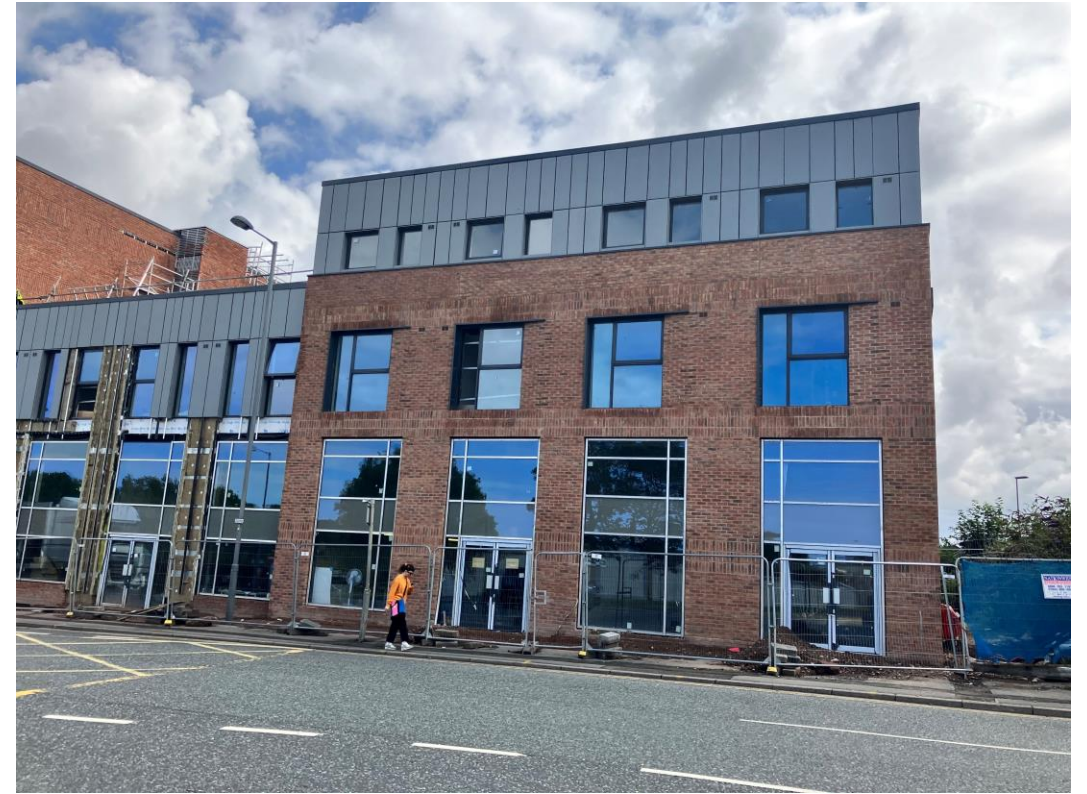
Commercial Block - Curtain walling
