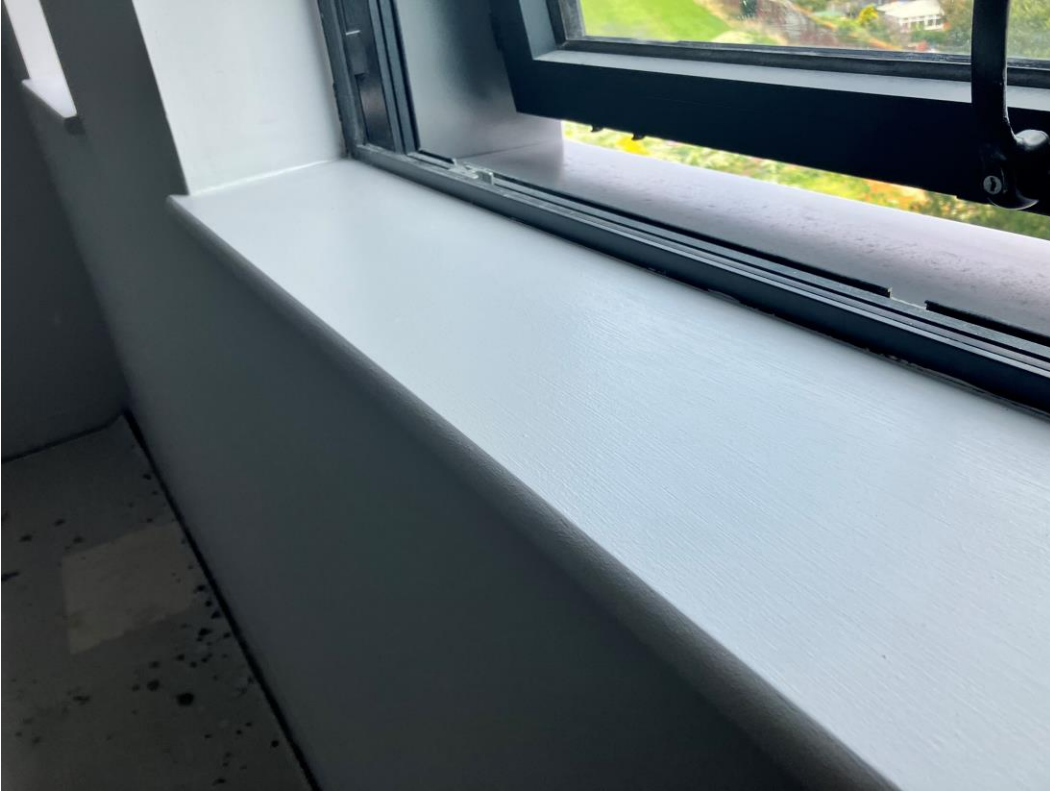
Residential Block – MDF Window boards
