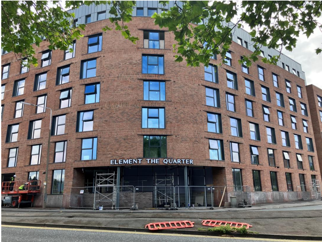
Brunswick Road – Building signage complete
