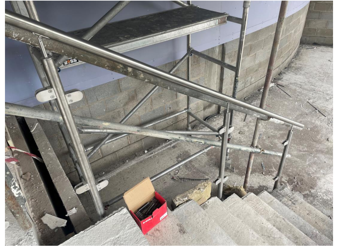
Main Entrance – Metal handrail installed
