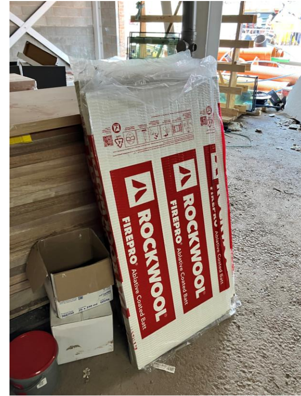
Material Storage – Rockwool Fire Batt
