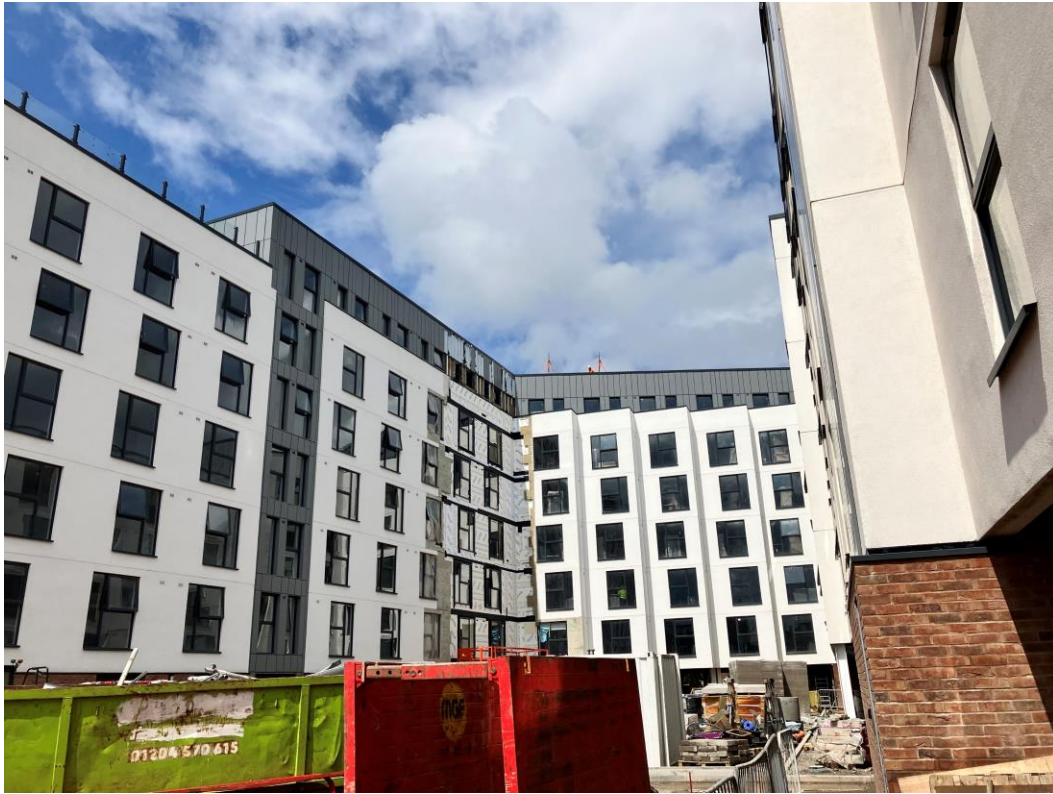
Residential Wing – Cladding installation nearing completion
