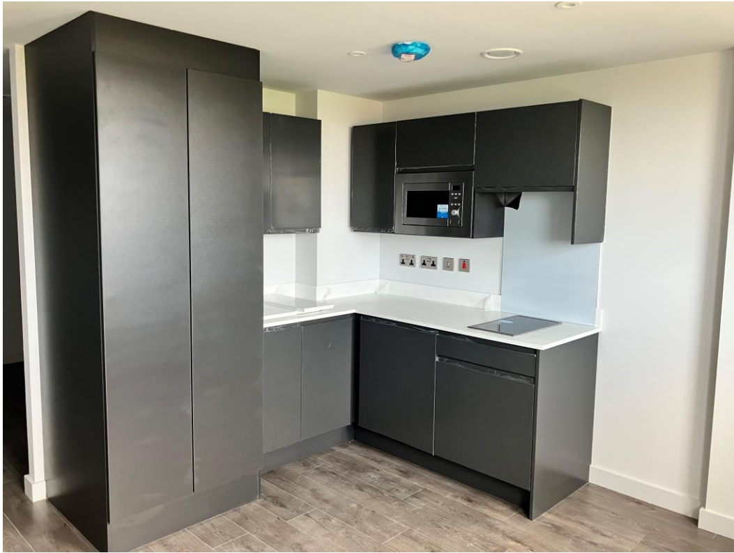
Residential Block – Kitchen installation
