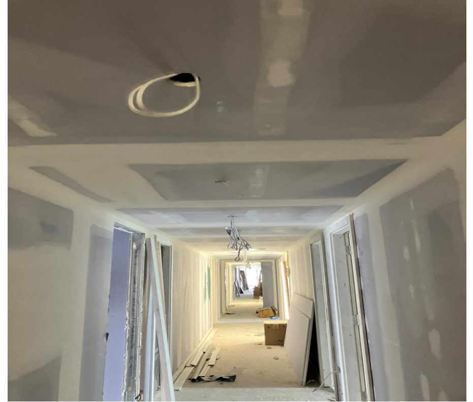
Residential Block – Corridor ceilings & walls tape & jointed
