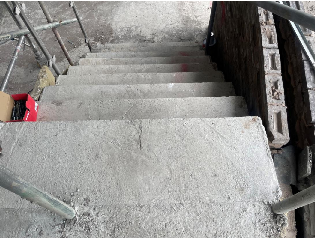
Main Entrance – Concrete staircase formed
