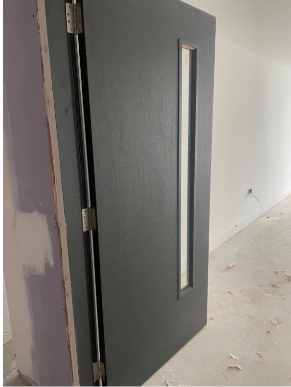
Ground Floor – Doors installed
