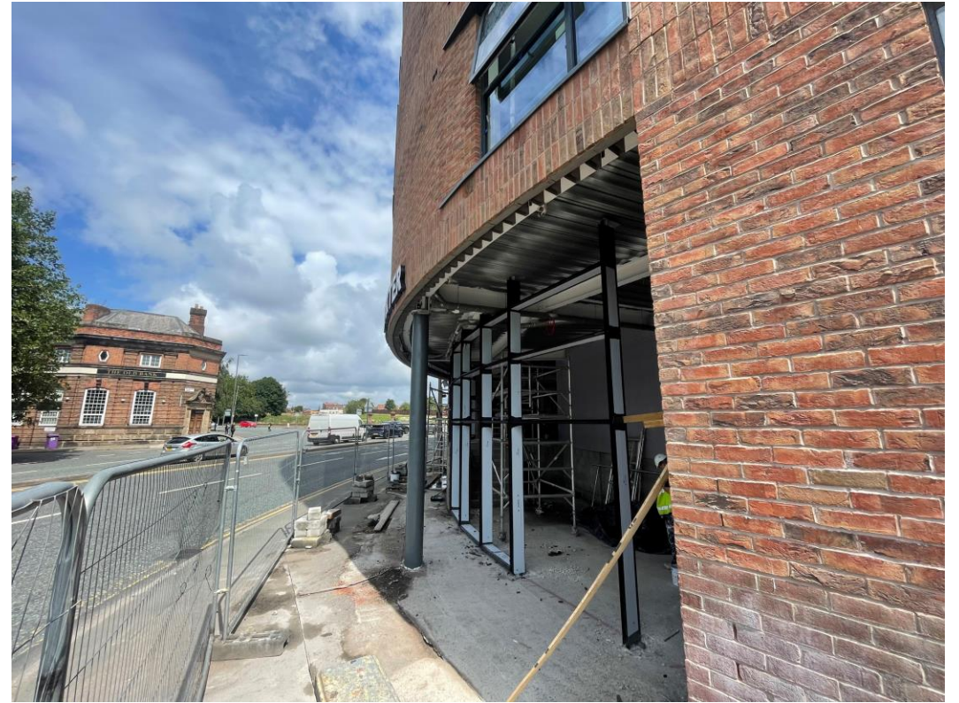
Main Entrance – Curtain wall installation
