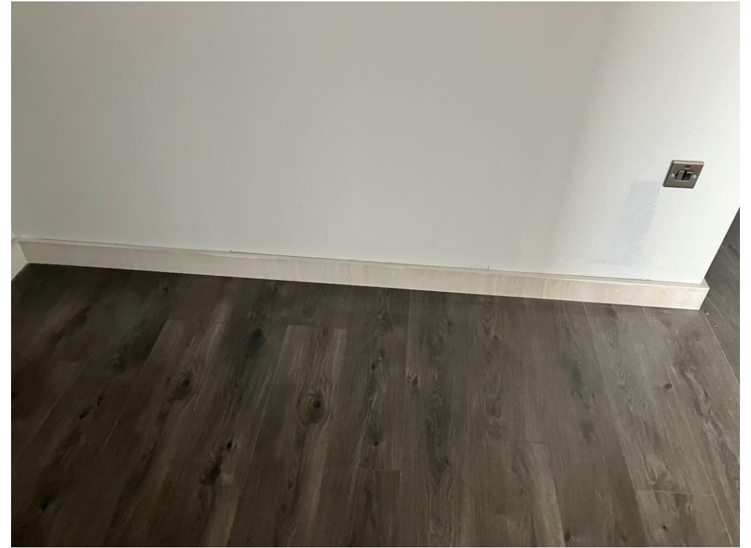
Residential Block – Skirting installation on-going
