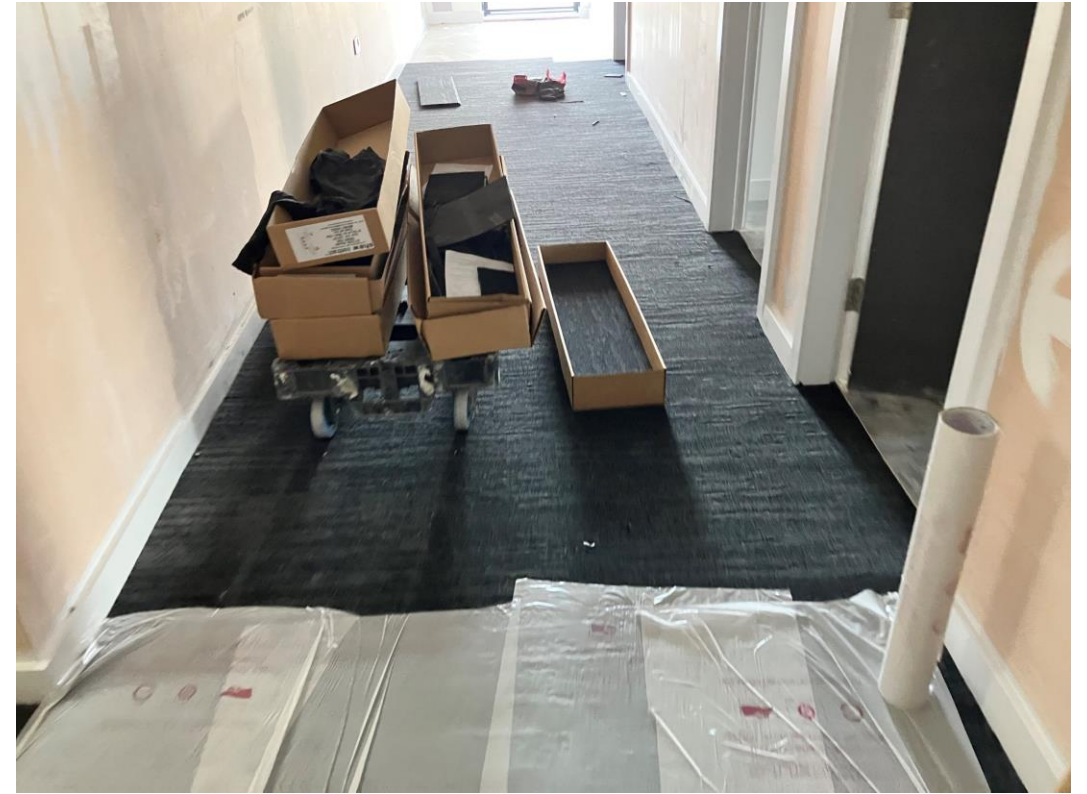
Material storage – Carpet Tiles
