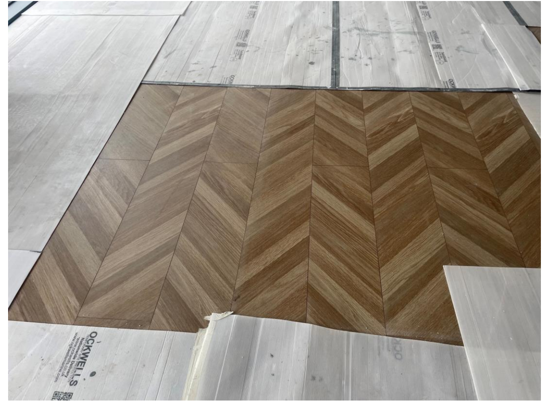
Ground Floor Games / Lounge – Laminate flooring installation complete
