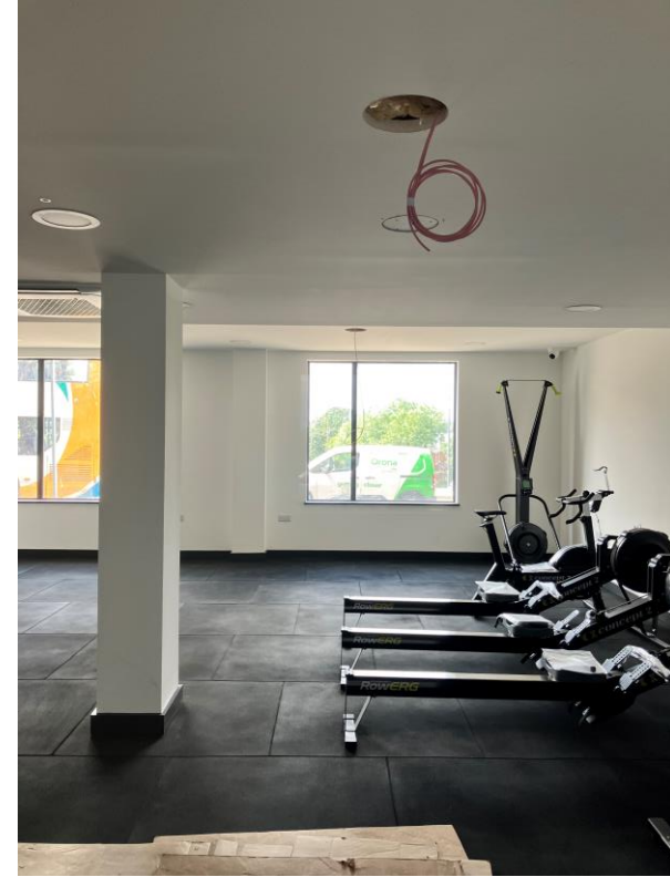
Ground Floor – Gym equipment
