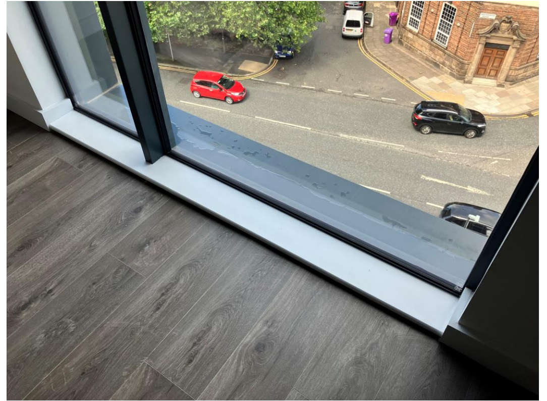
Residential Block – Window board installed & decorated
