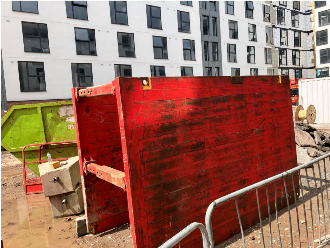
Excavation shoring boxes
