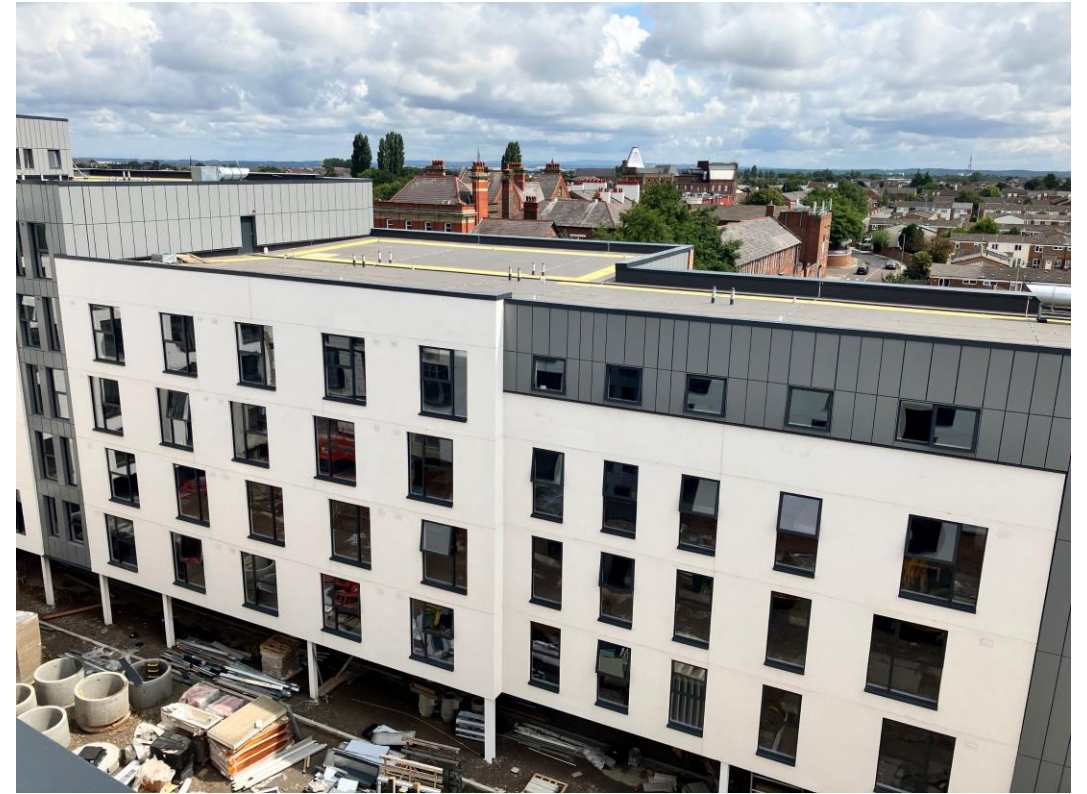
Student Block – Cladding complete
