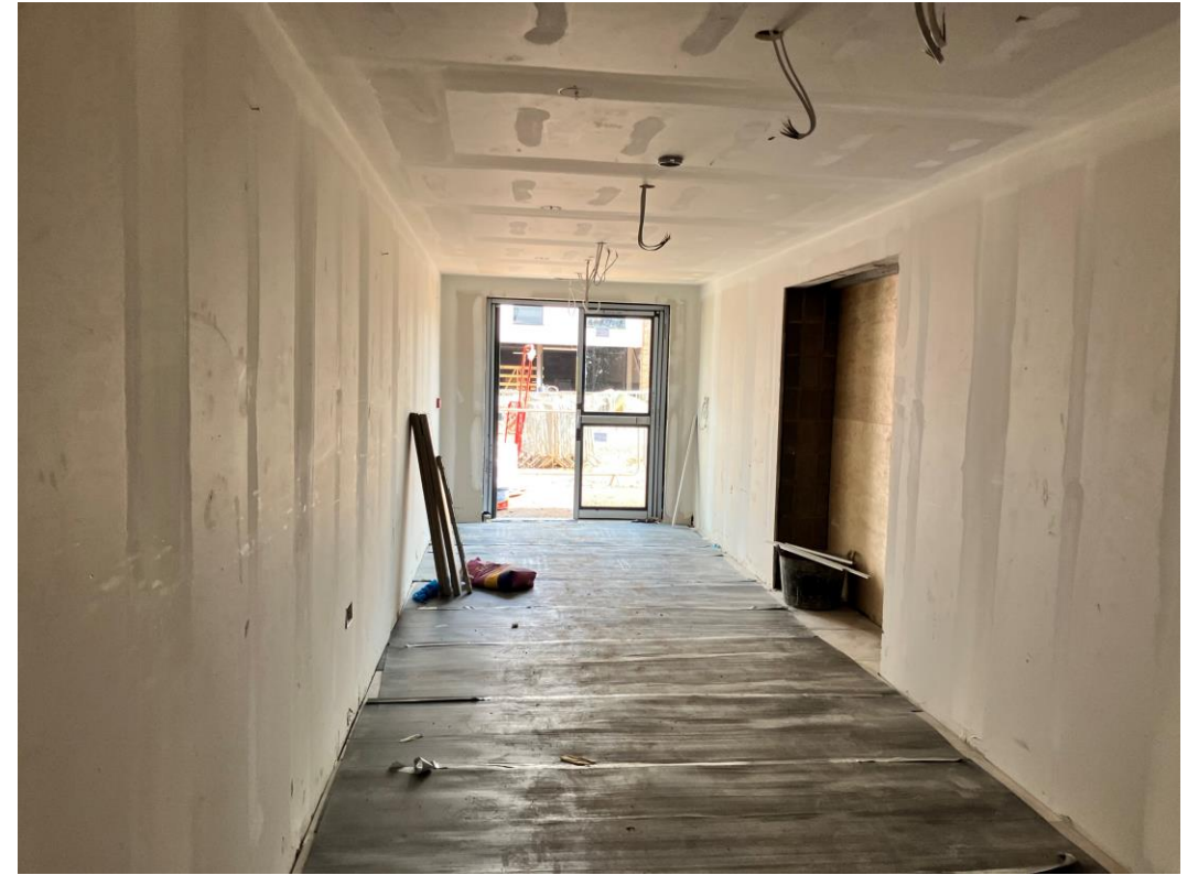
Ground Floor – Tape & jointing to Lobby walls & ceilings
