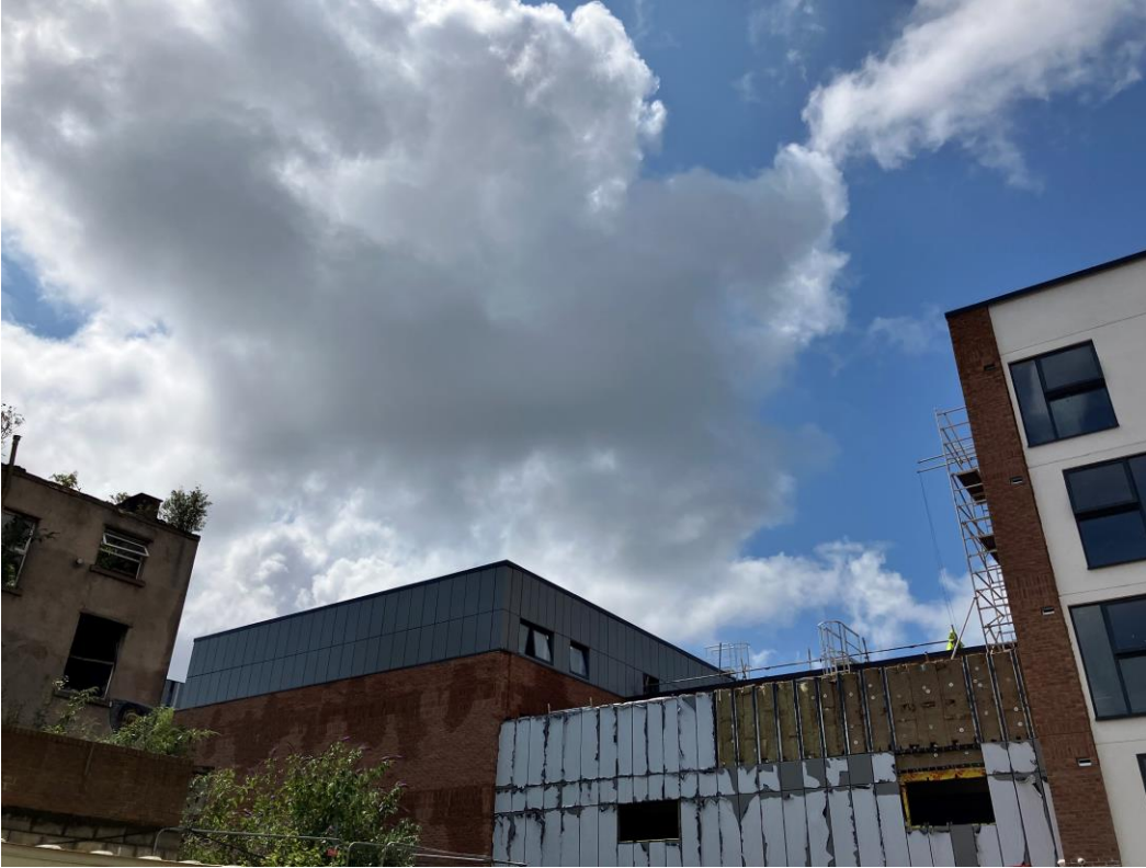
Commercial Zone – Rainscreen cladding on-going
