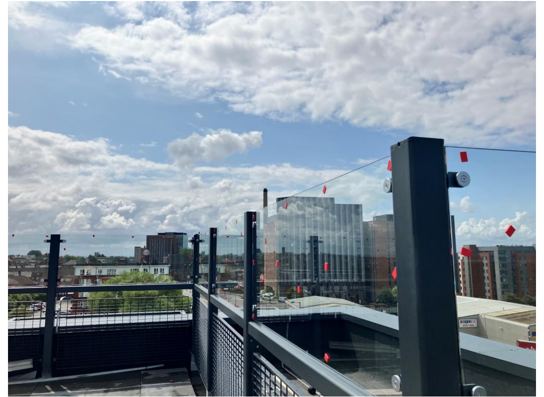
Residential Wing – Glazed balustrade installation nearing completion
