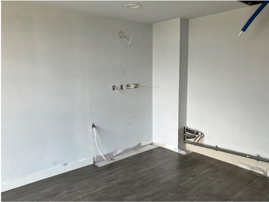
Residential Block – Decoration works on-going
