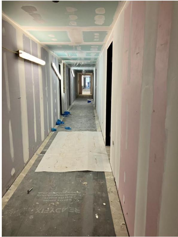
Ground Floor – Tape & jointing to Corridor walls & ceilings
