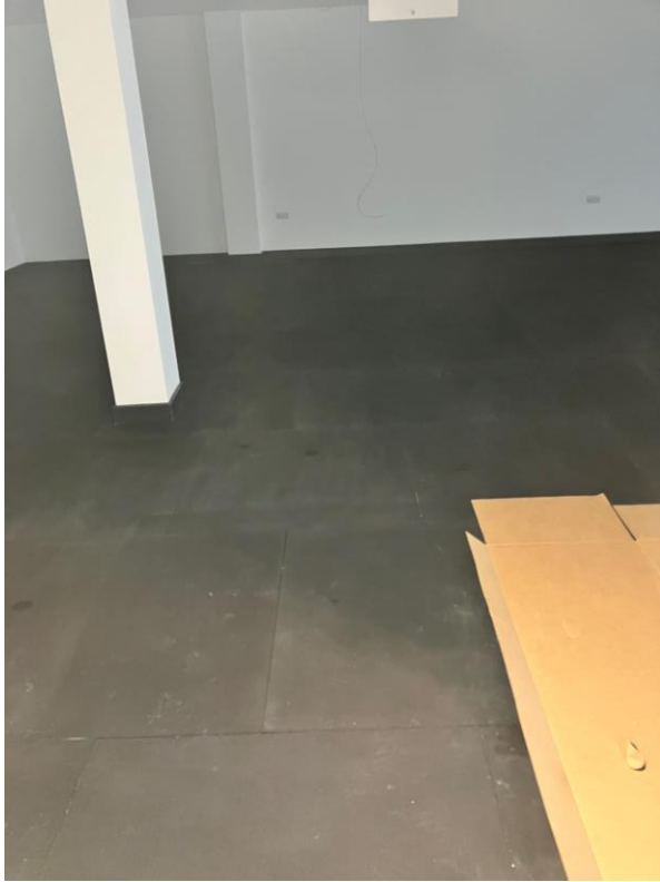
Ground Floor – Rubber gym flooring in place
