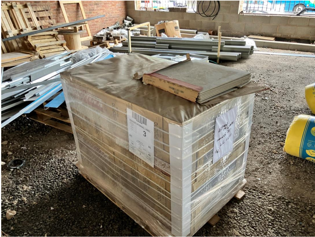
Material storage – Wall & Floor Tiles
