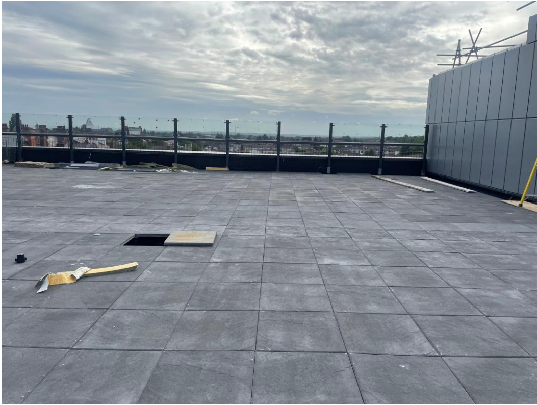
Residential Block – Paving
