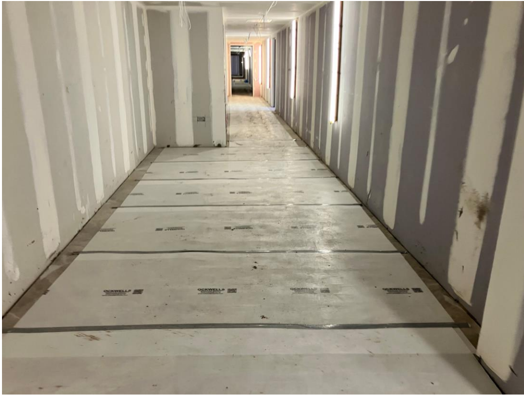
Ground Floor– Floor tiling on-going. Protection in place
