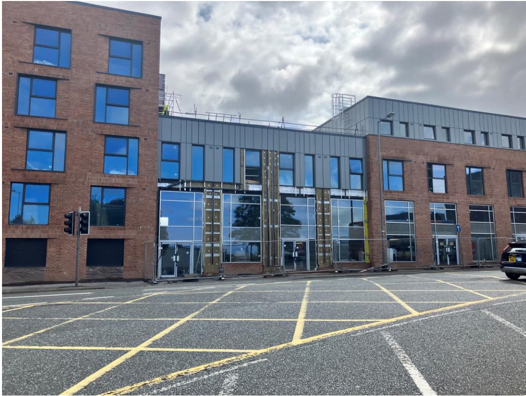
Commercial Block - Curtain walling
