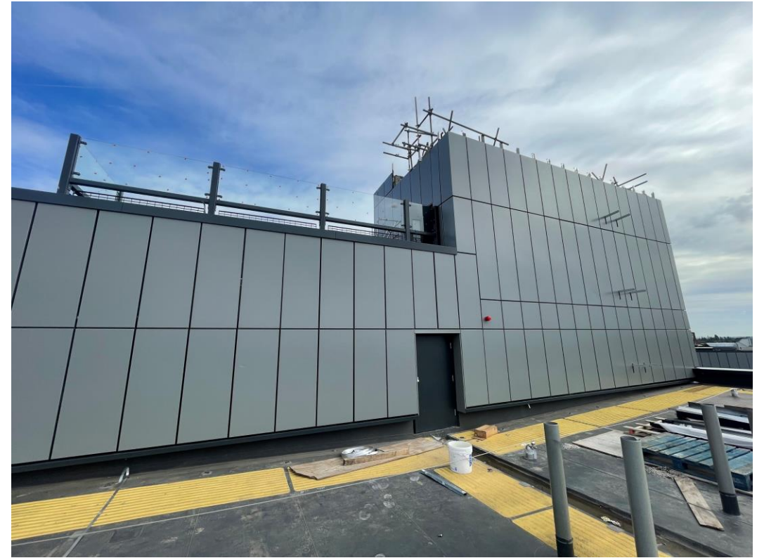
Residential Block – Rainscreen cladding
