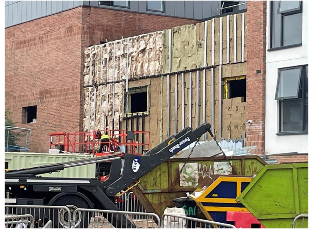
Commercial Zone – Rainscreen cladding installation commenced
