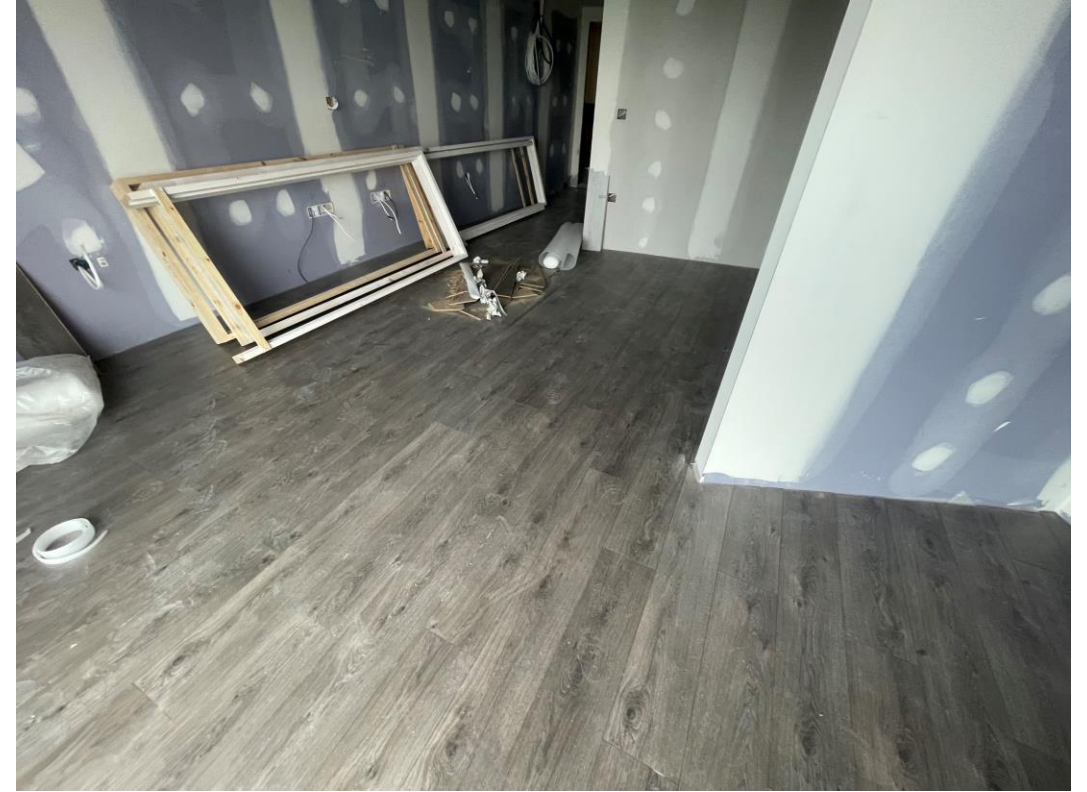
Residential Block – Laminate installation on-going
