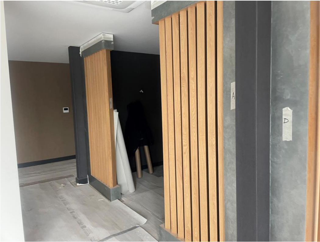
Ground Floor – Slattered Timber detail
