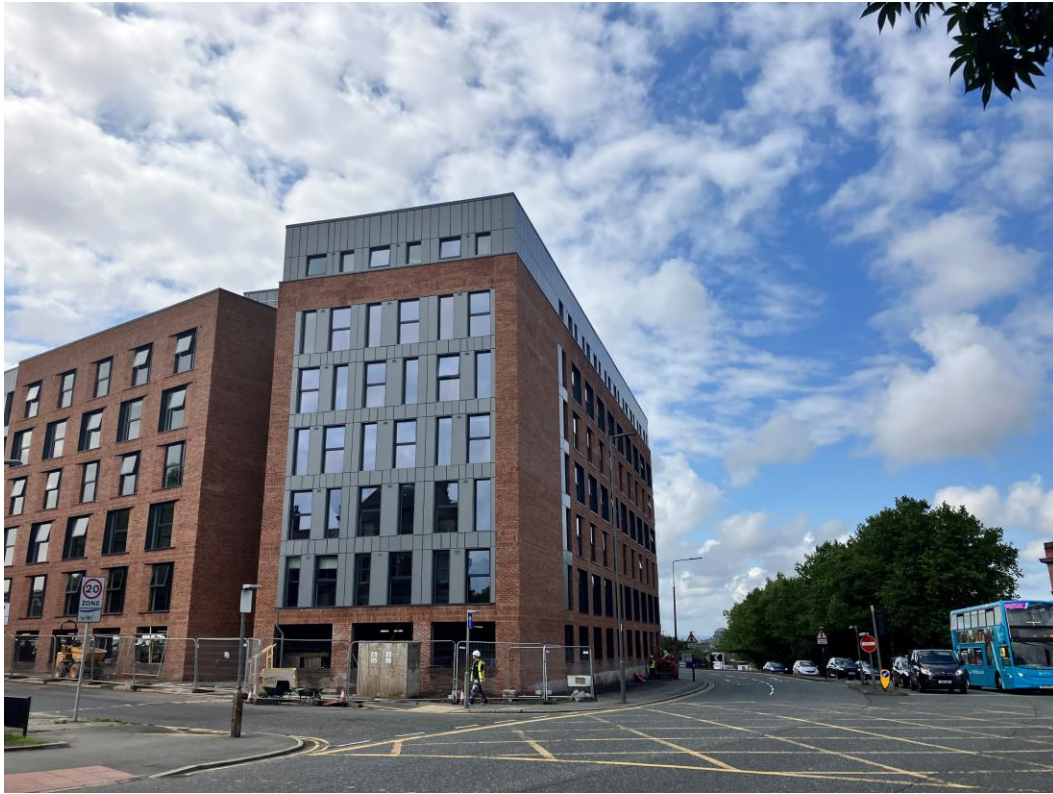
West Derby Road - Site view
