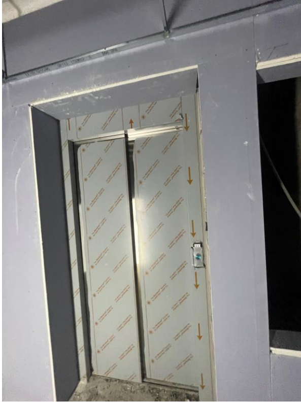
Student Block – Boarding of lift walls on-going
