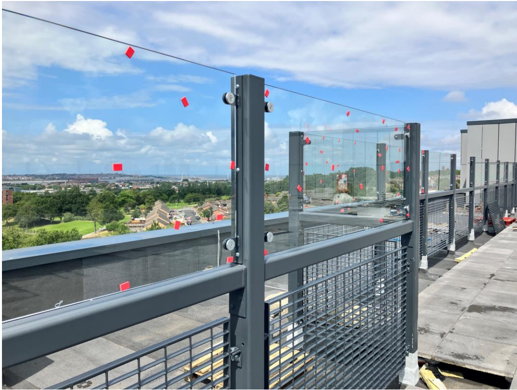
Residential Wing – Glazed balustrade installation nearing completion
