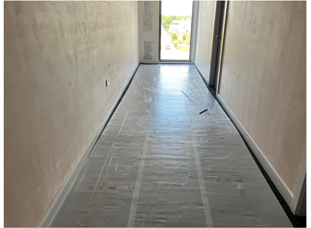
Student Block – Corridor carpet tiles
