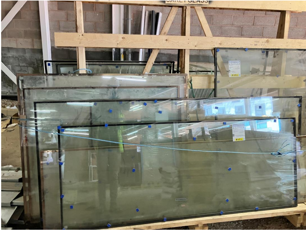
Material storage – Glazing units
