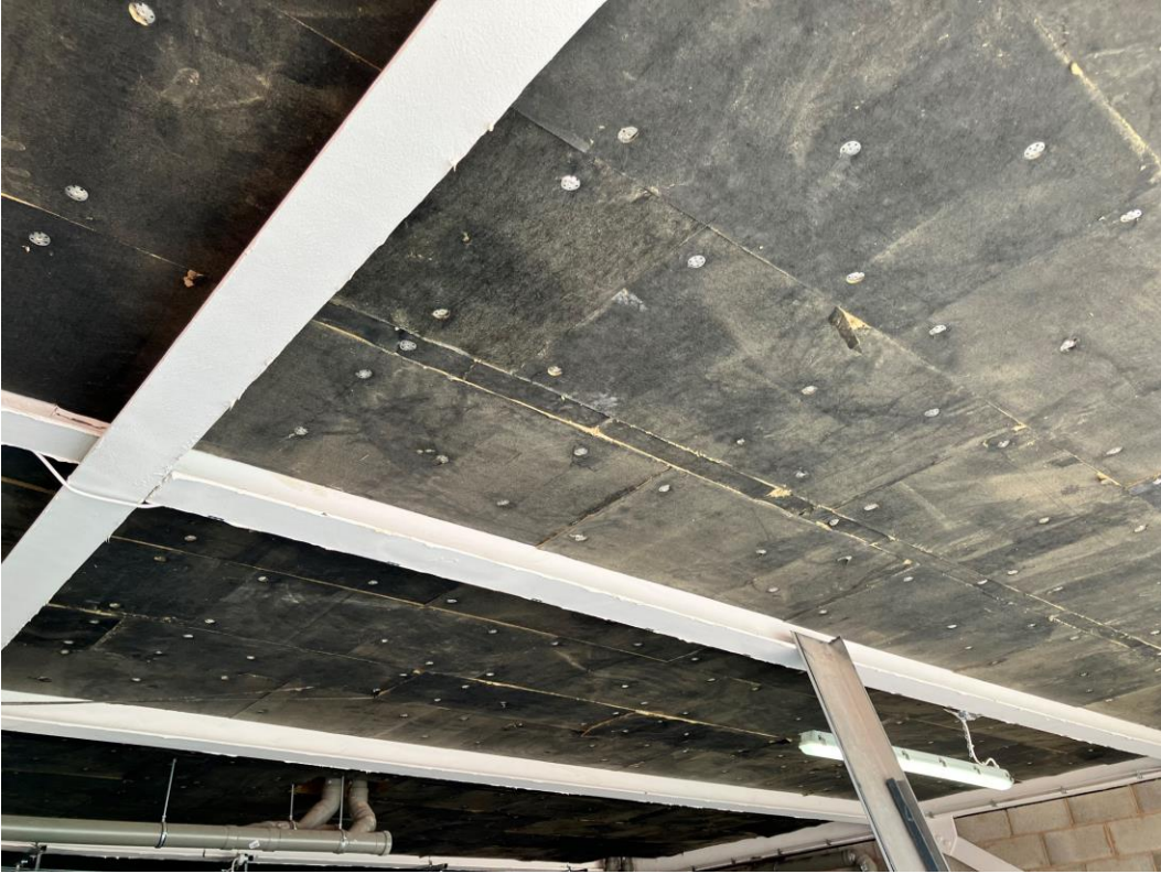
Ceiling soffit insulation detail installed
