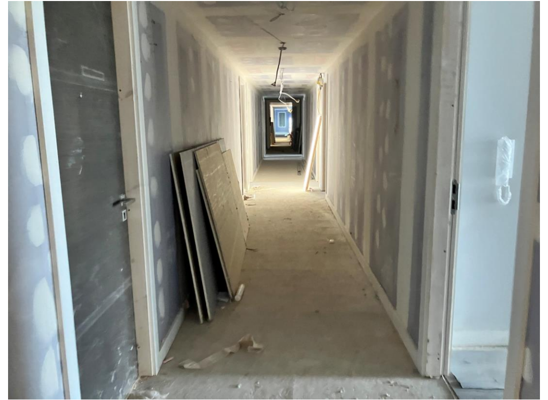
Residential Block – Corridor walls & ceilings tape & jointed
