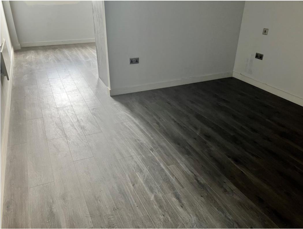
Residential Block – Laminate flooring installed
