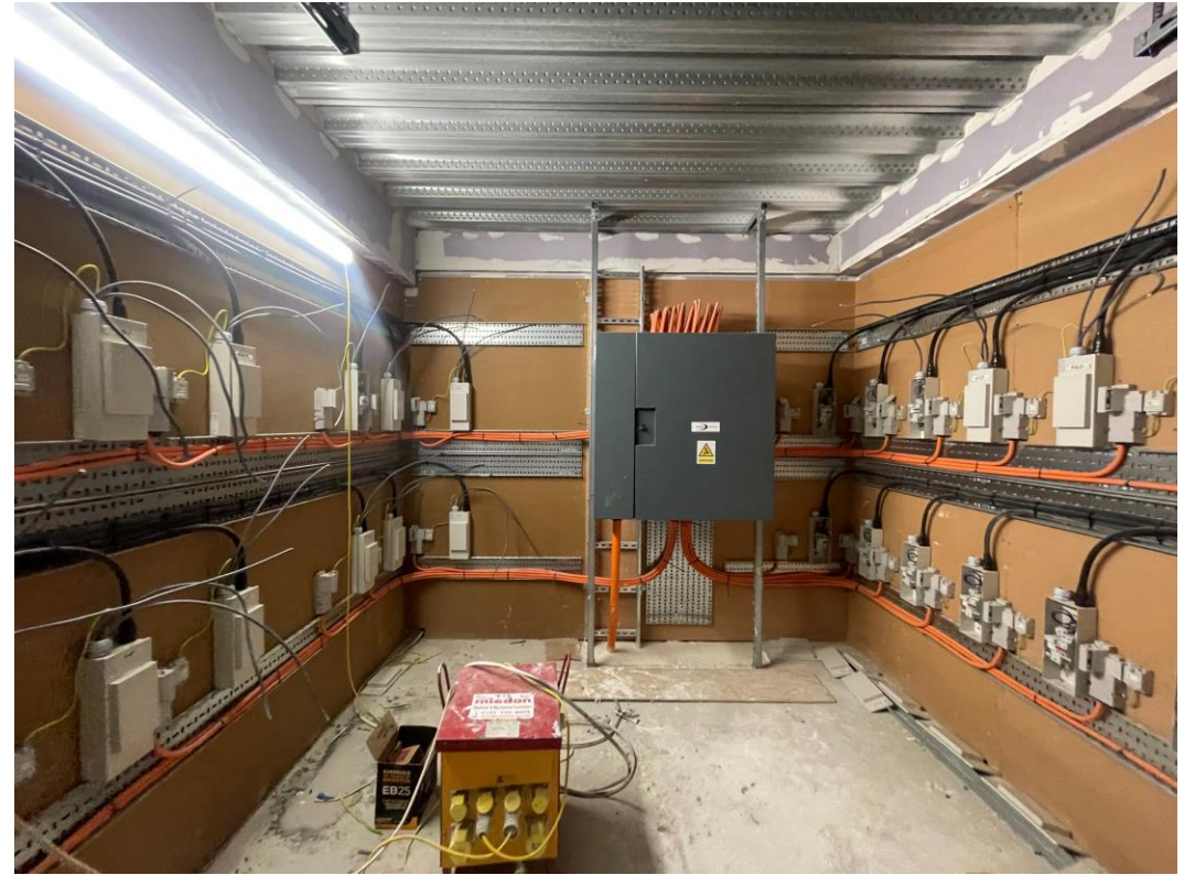
Residential Block – Apartment metres installation
