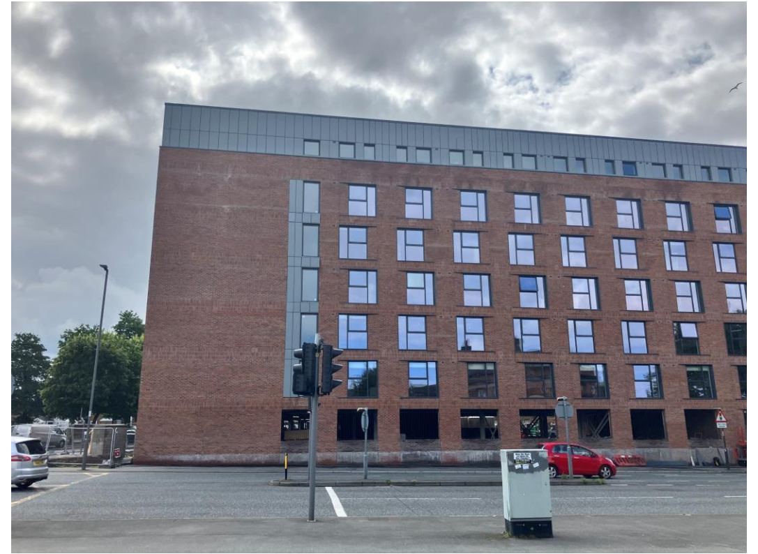
West Derby Road - Site view
