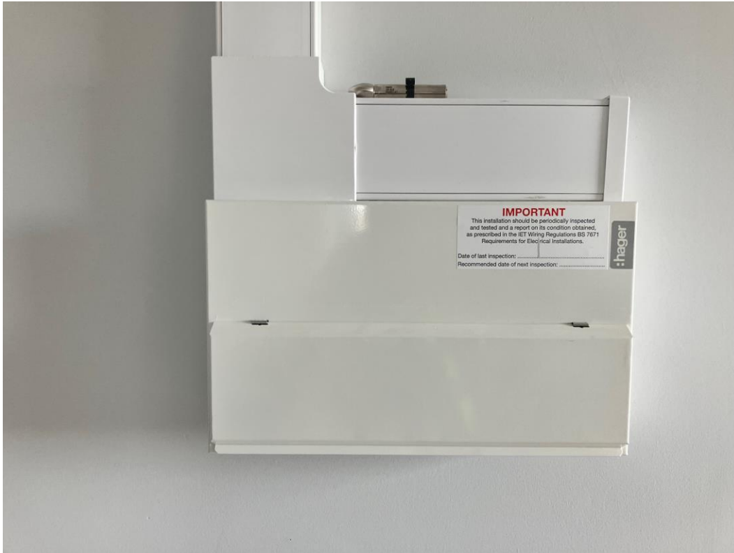
Residential Wing – Kitchen installation
