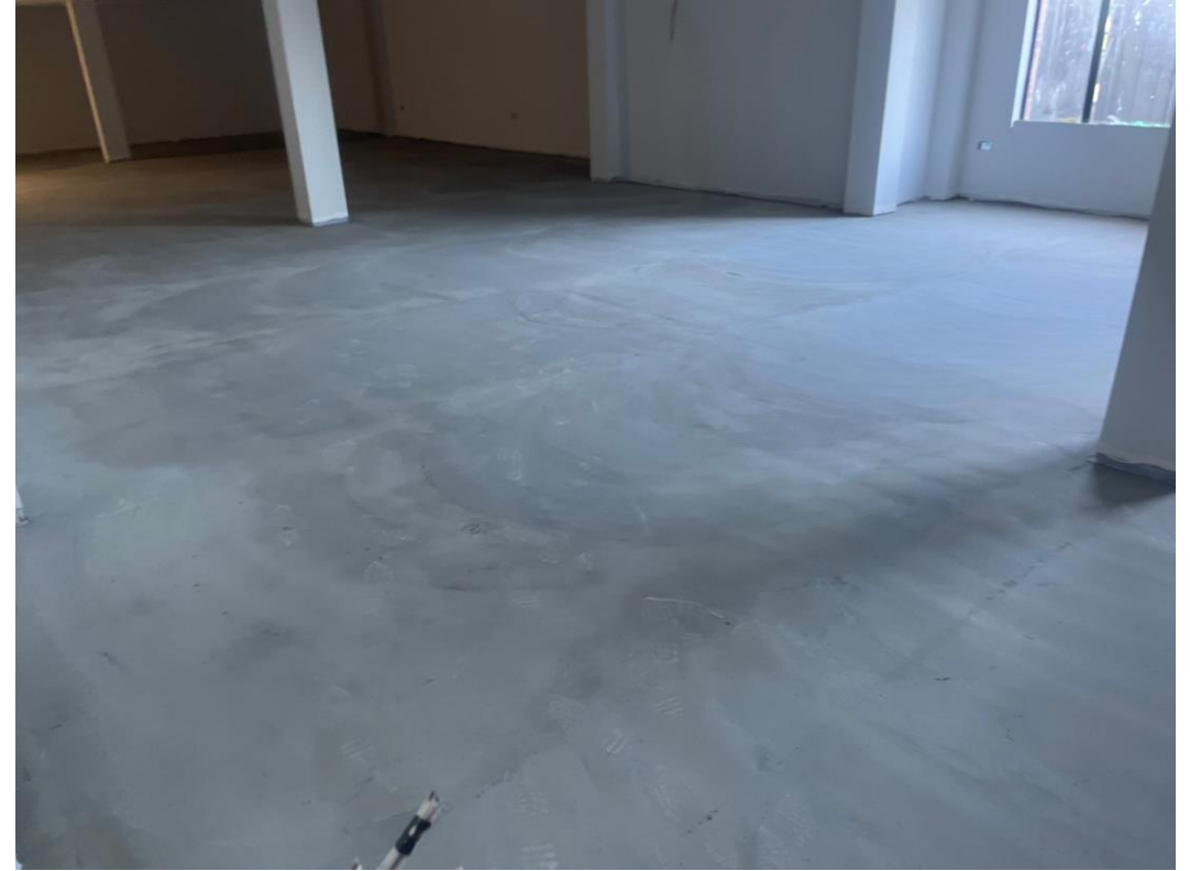
Ground Floor – Latex screed
