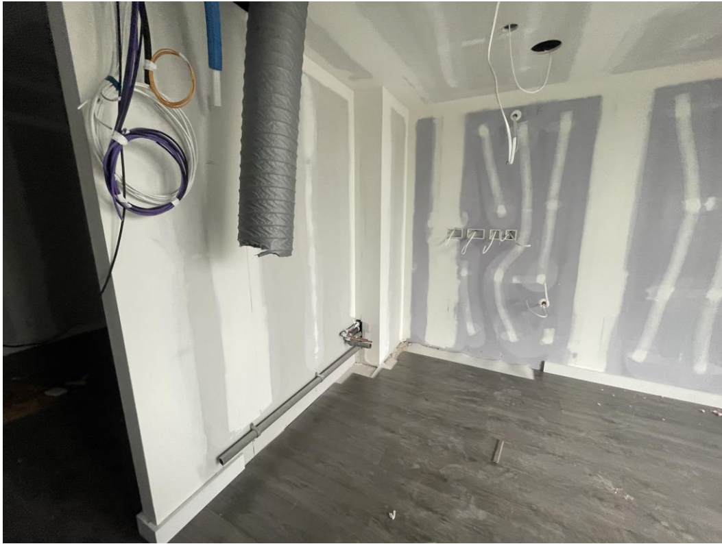
Residential Block – Laminate flooring installed
