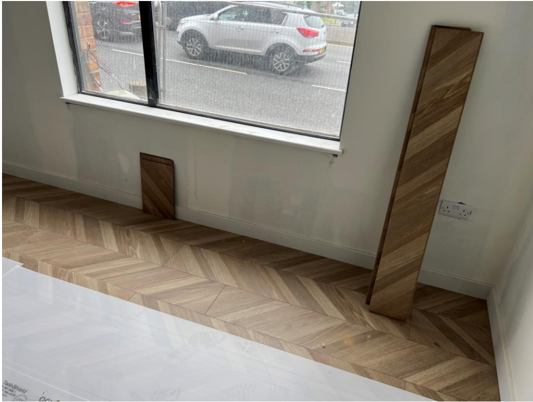
Ground Floor– Laminate flooring installation commenced
