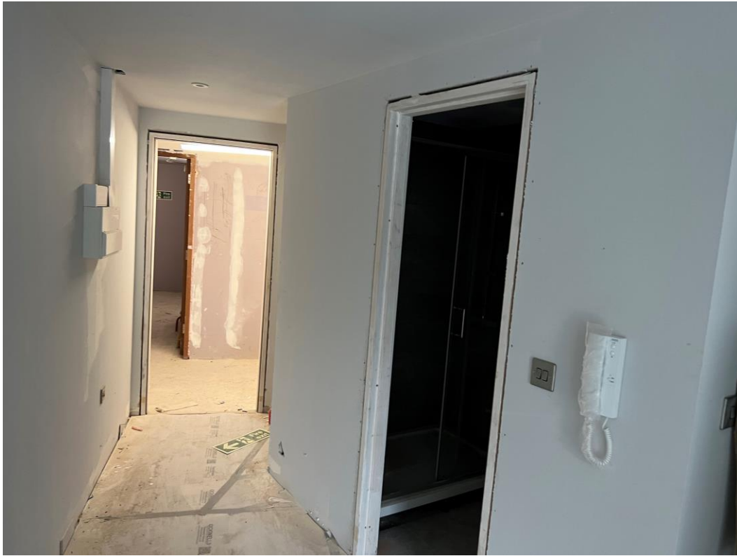
Residential Block – Decoration works on-going
