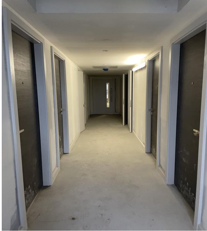
Residential Block – 2 nd coat decoration complete
