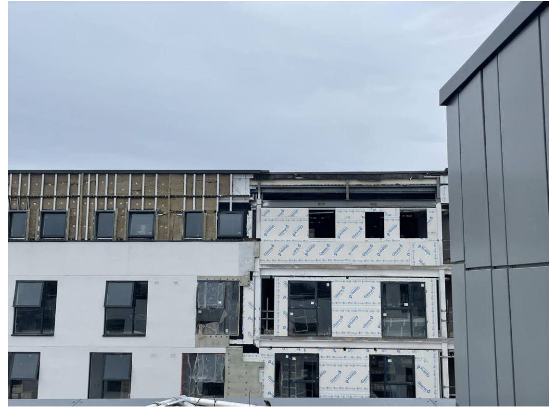
Rainscreen cladding installation nearing completion
