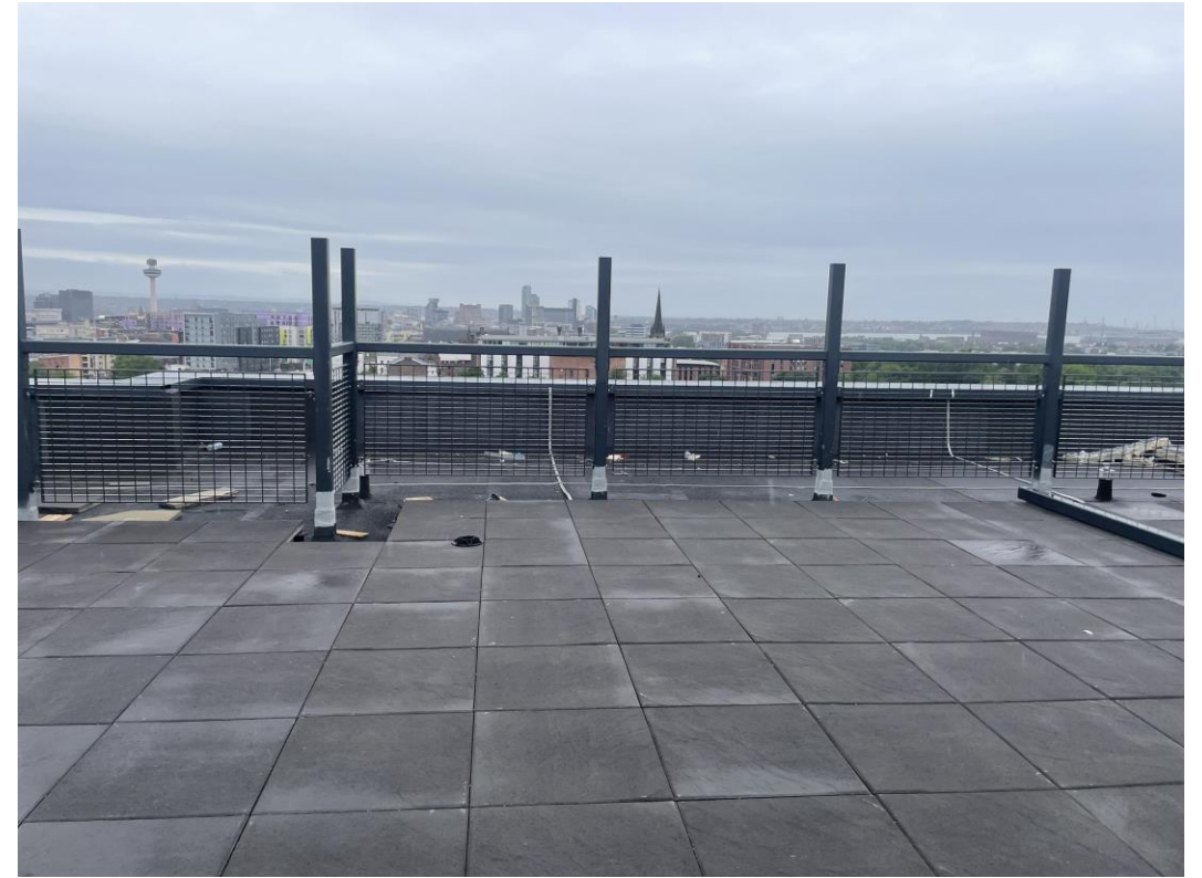
Residential Wing – Paving installation on-going
