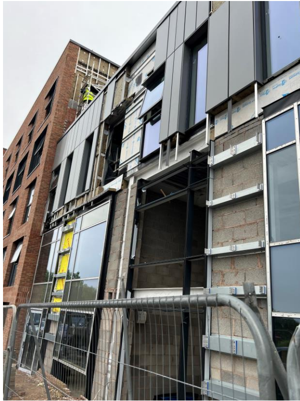
Commercial Units – Cladding nearing completion
