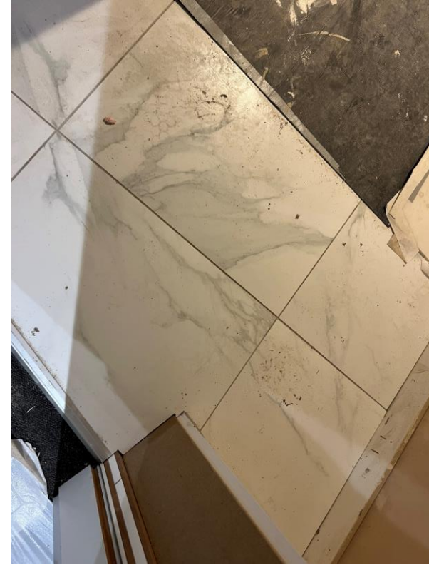
Residential Block – Lift lobby tiled flooring
