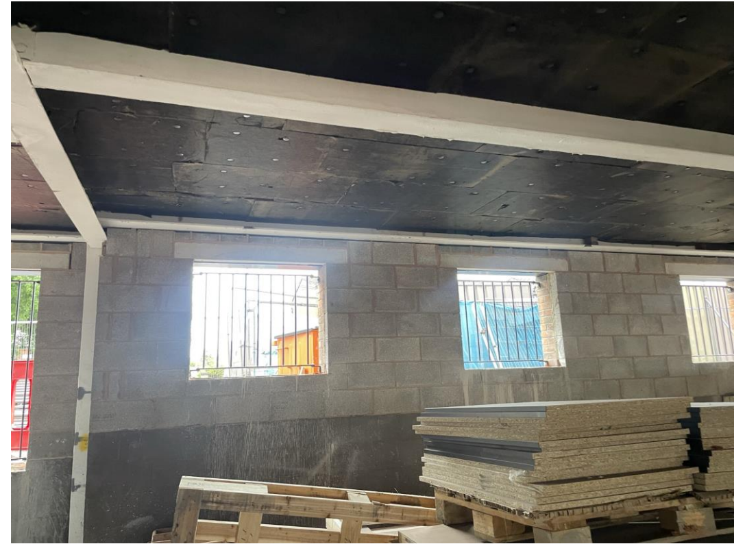
Under croft Car Park – Railings installed
