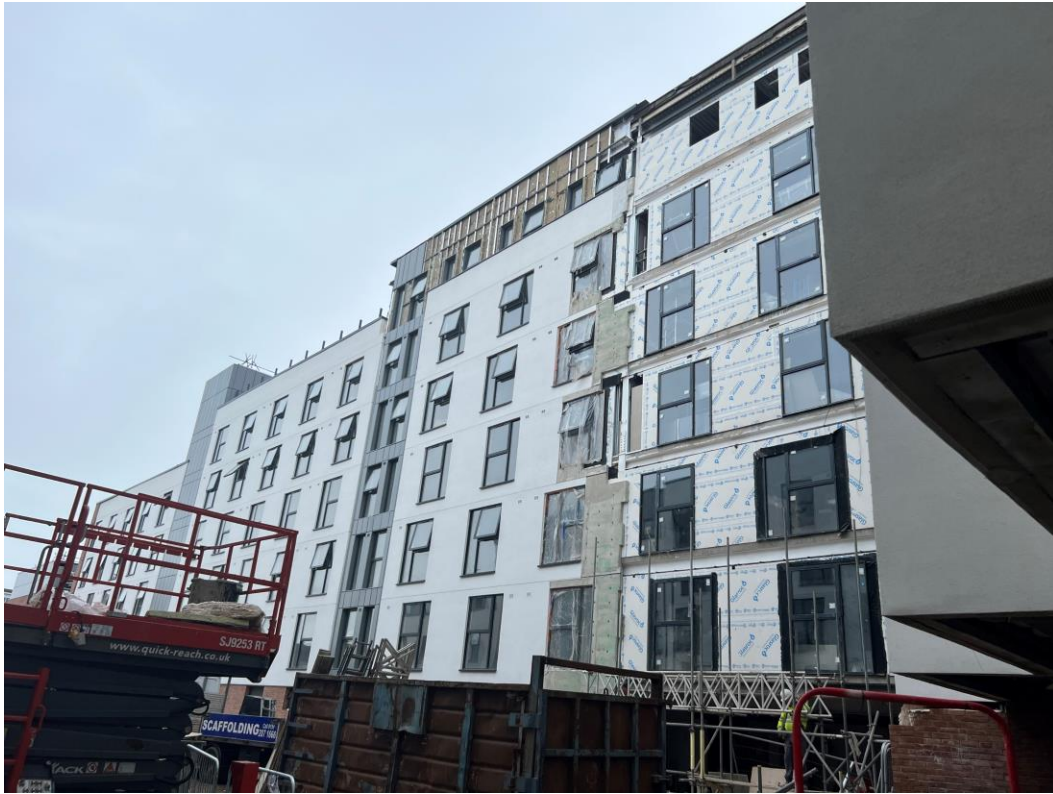
Residential Block – Removal of hoist lift nearing completion
