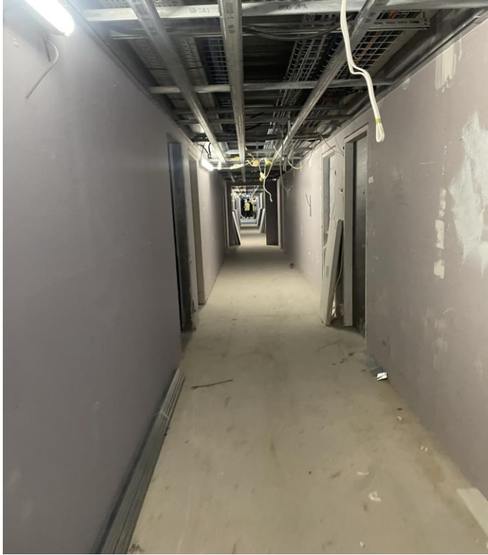
Residential Block – Corridor walls boarded
