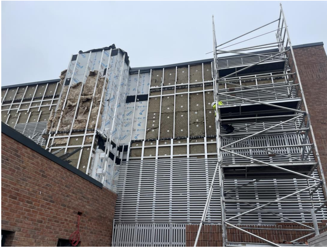
Residential - Brick slip installation on-going
