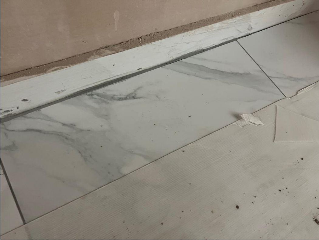
Residential Block – Lift lobby tiled flooring
