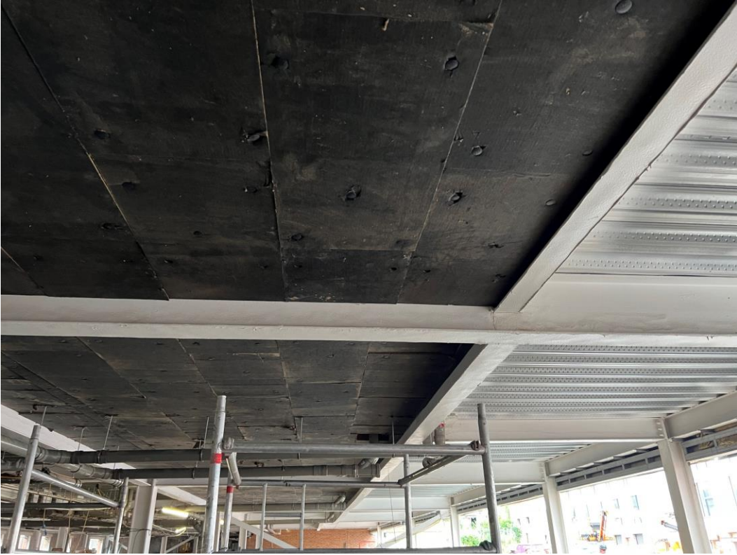
Ceiling soffit insulation detail installed
