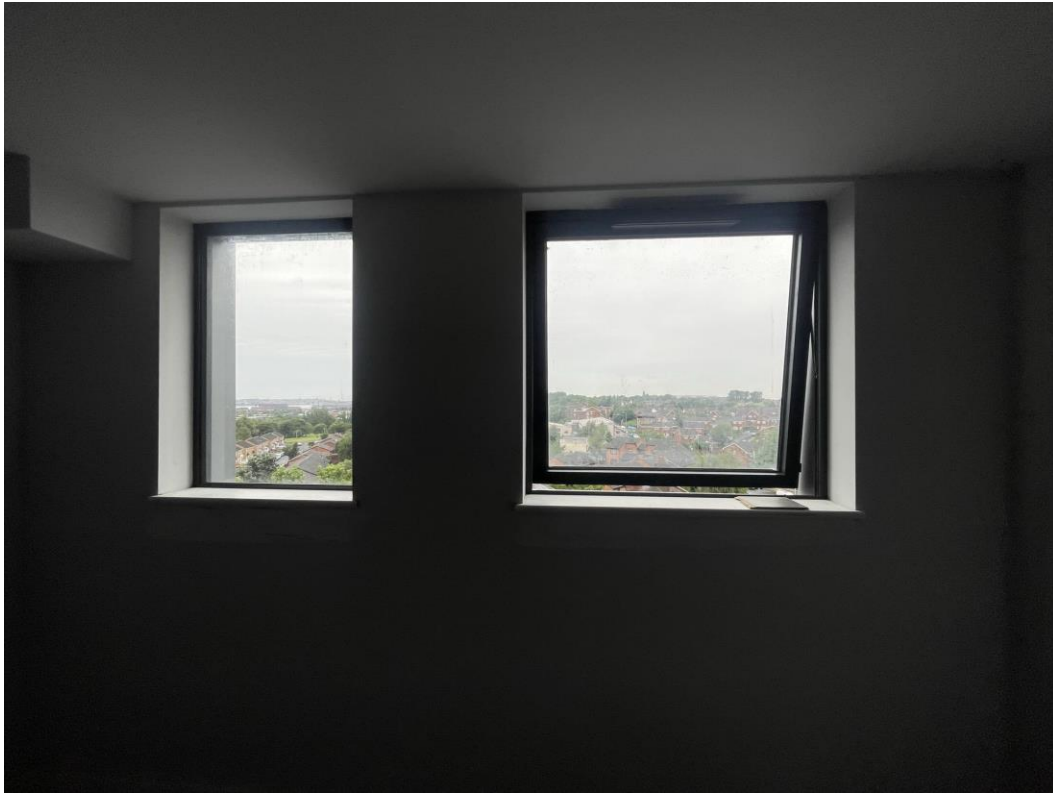
Residential Block – MDF Window boards
