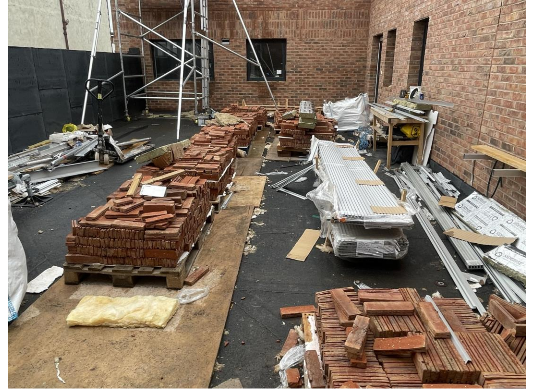
Materials Stored – Brick Slip
