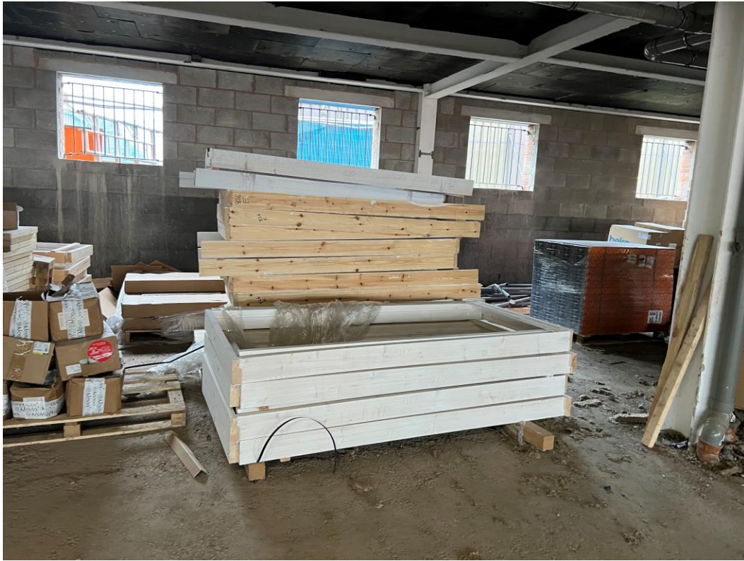
Material storage – Door casings
