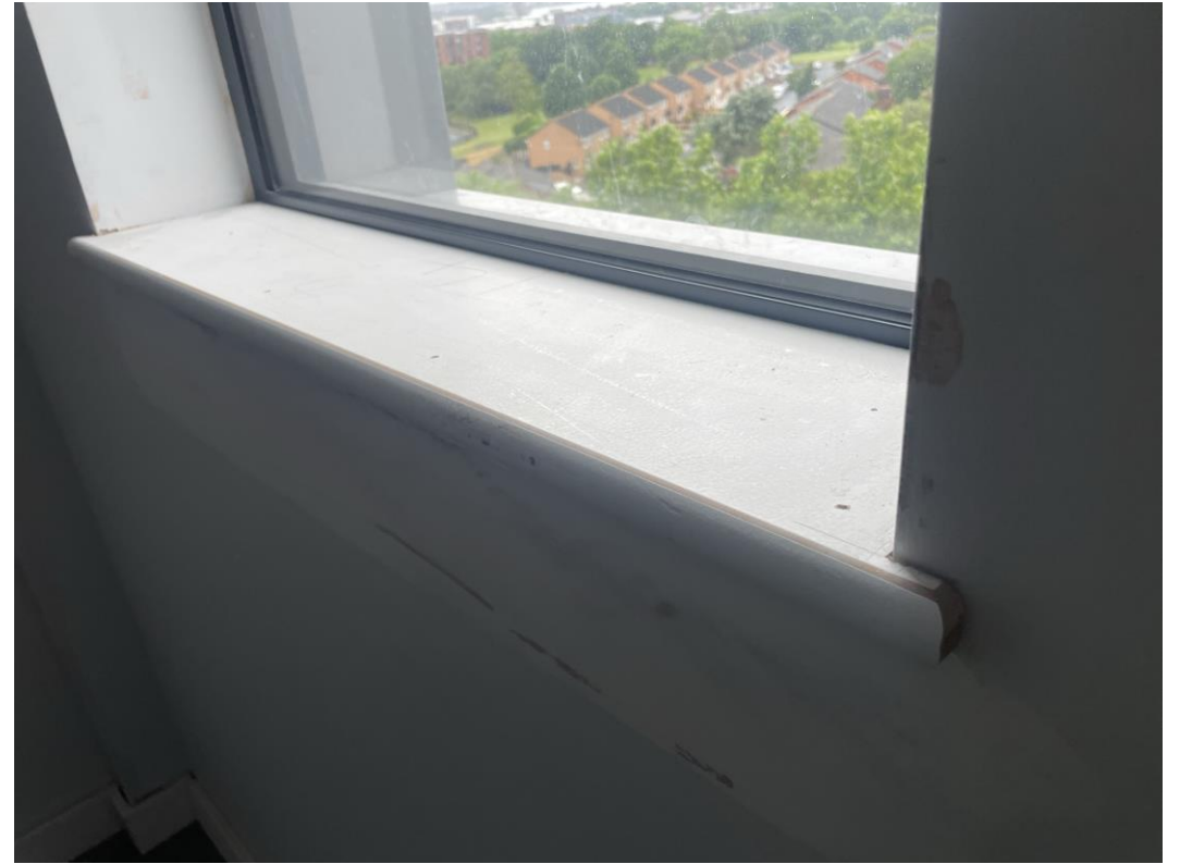
Residential Block – MDF Window boards
