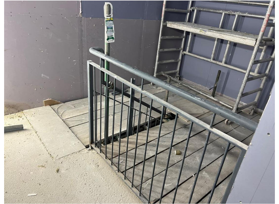
Student Block – Temporary working platform
