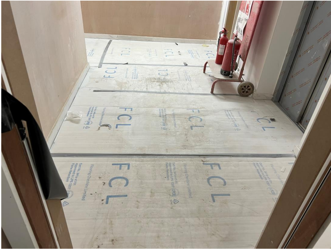
Student Block – Lift Lobby floor tiled
