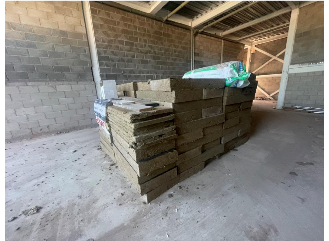
Materials Stored – Soffit insulation
