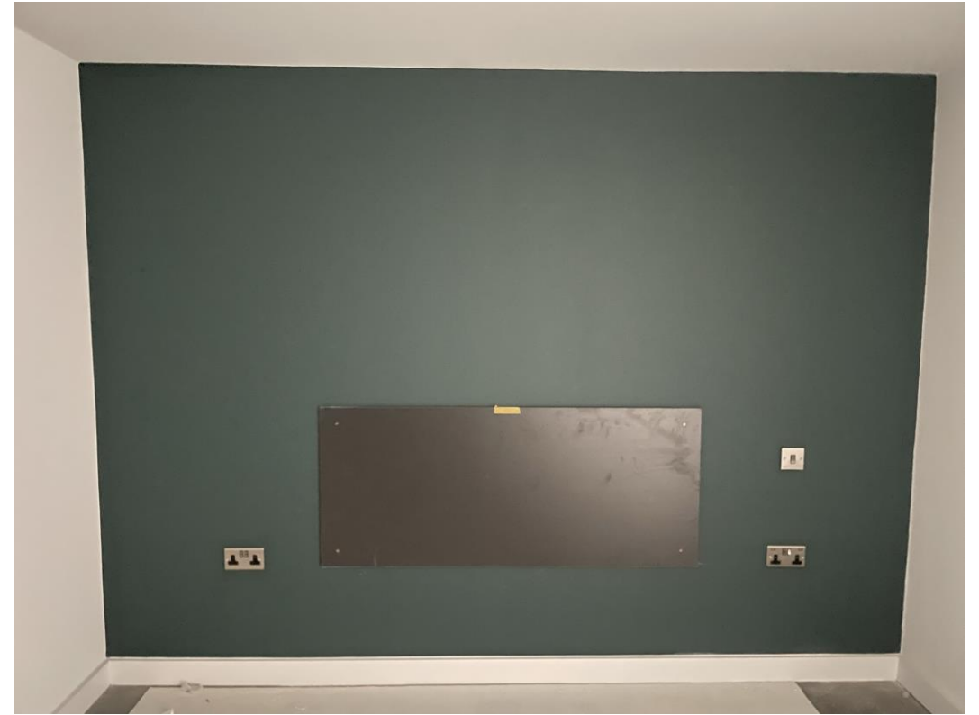
Residential Block – Bed head-board in place
