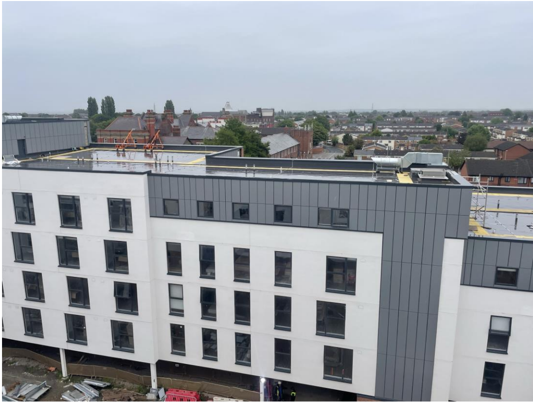
Student Wing – Rainscreen cladding complete
