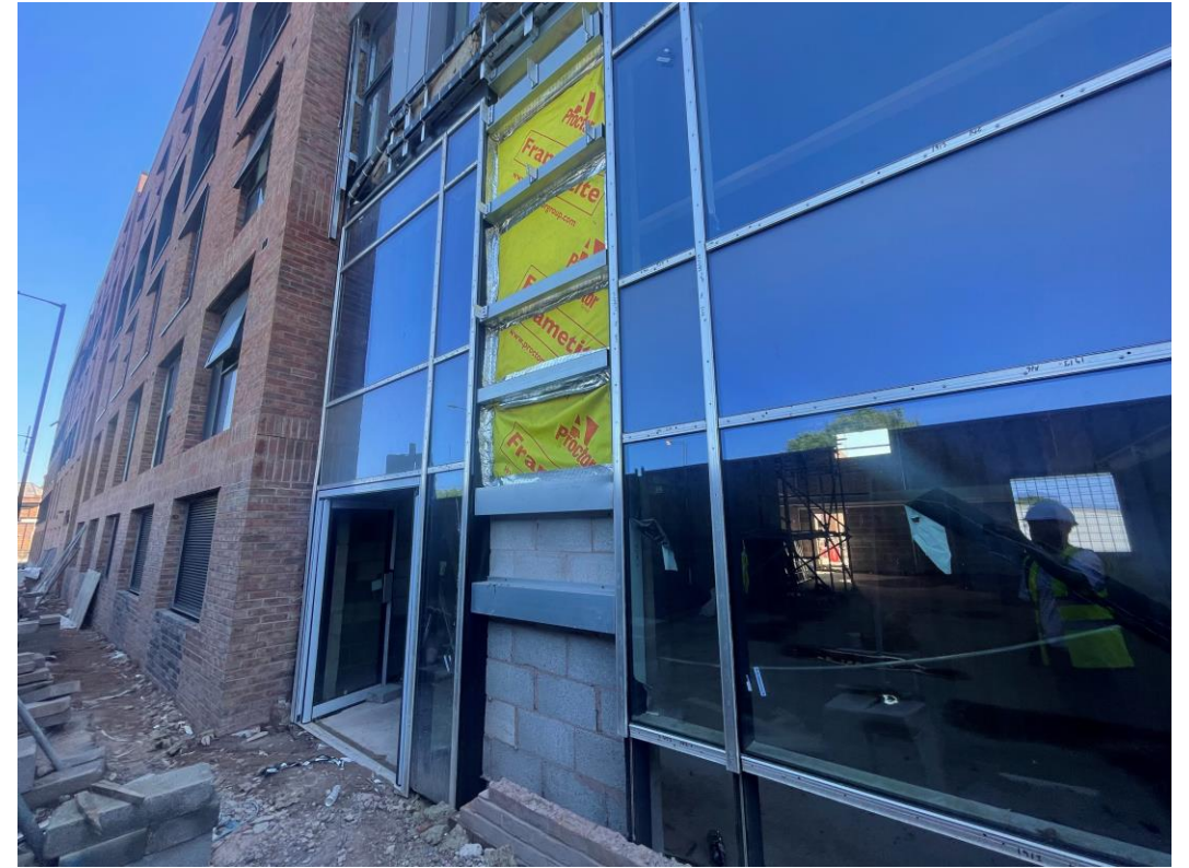
Commercial Block - Curtain walling
