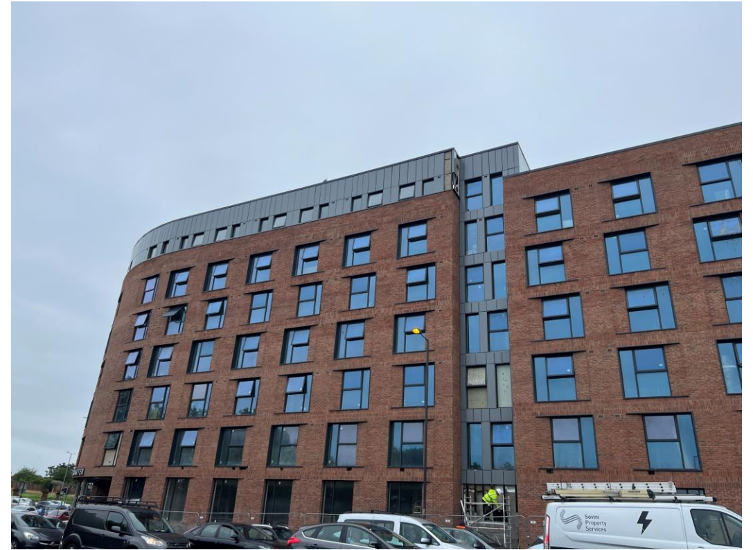
West Derby Road - Site view
