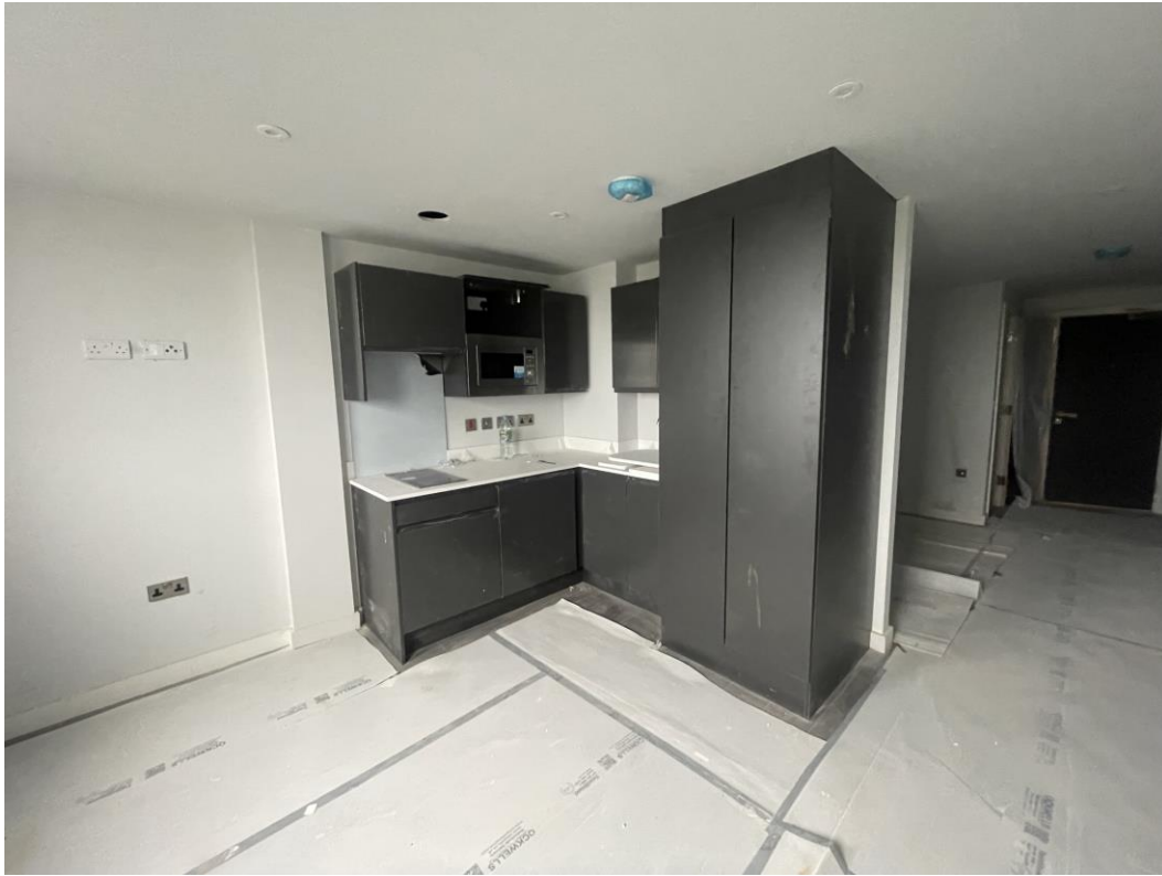
Residential Wing – Kitchen installation
