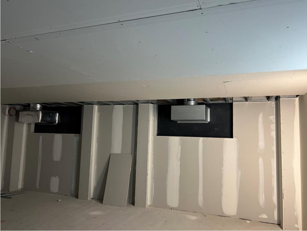
Ground Floor– Tape & Jointing
