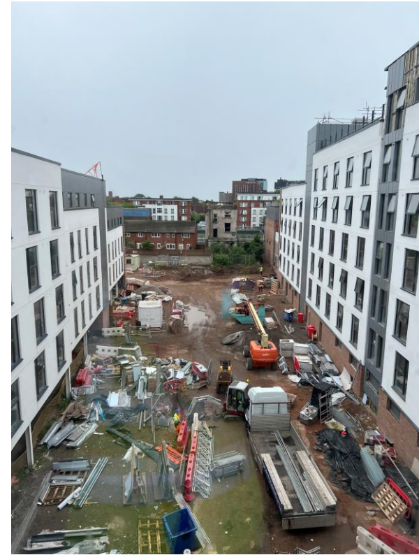
Residential Block – Site view
