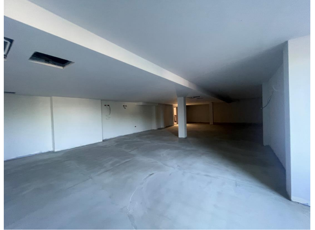
Ground Floor– Latex screed & Wall & Ceiling decoration
