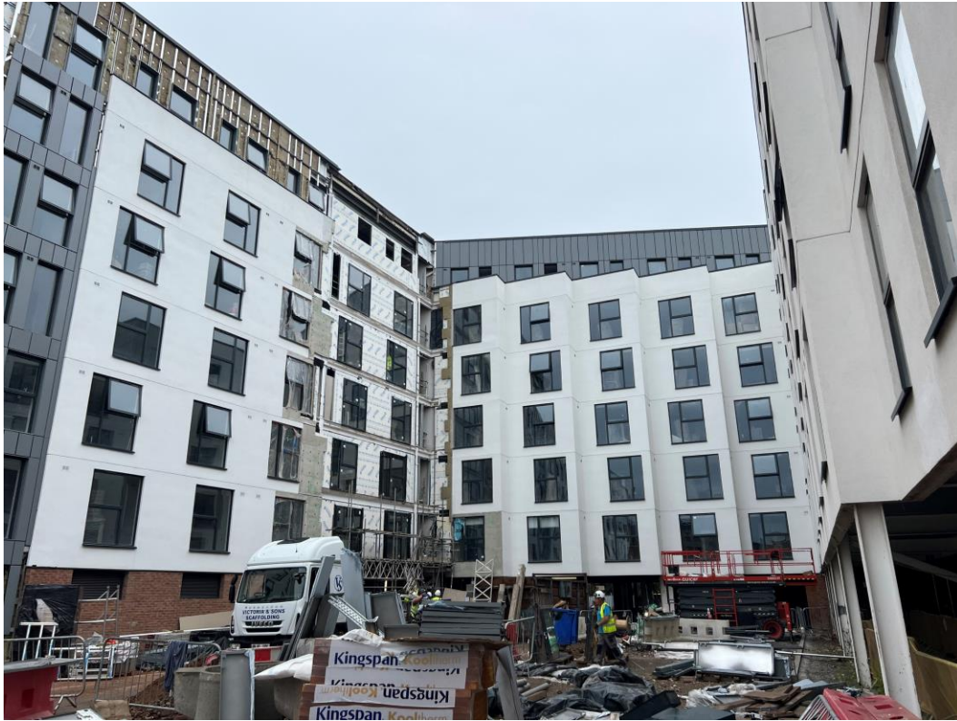
Residential Block – Viewed from site courtyard
