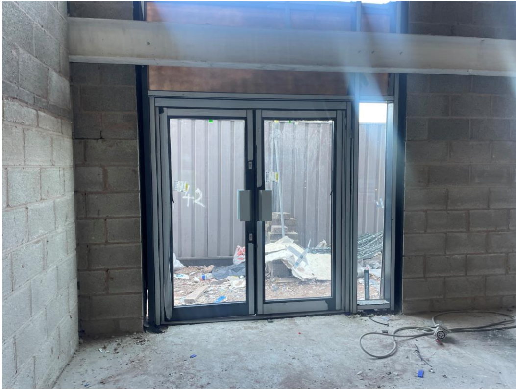
Commercial Block - Curtain walling
