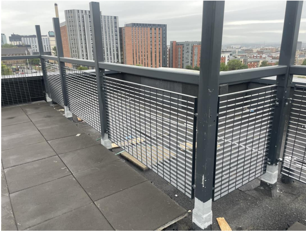
Residential Wing – Installation of metal balustrade on-going
