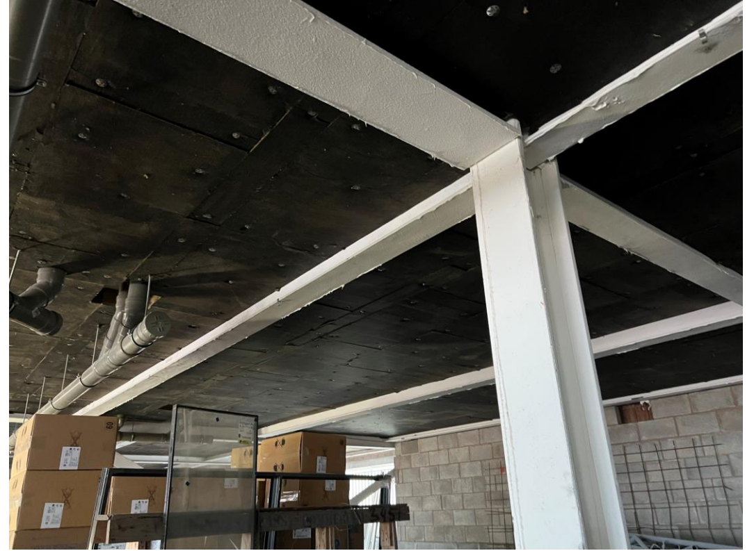
Ceiling soffit insulation detail installed
