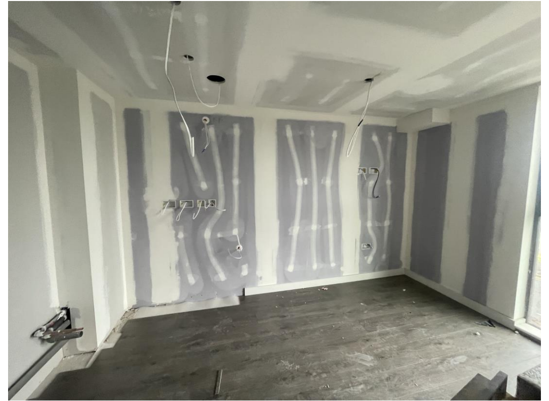
Residential Block – Laminate flooring installed
