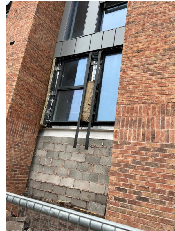
Window installation nearing completion
