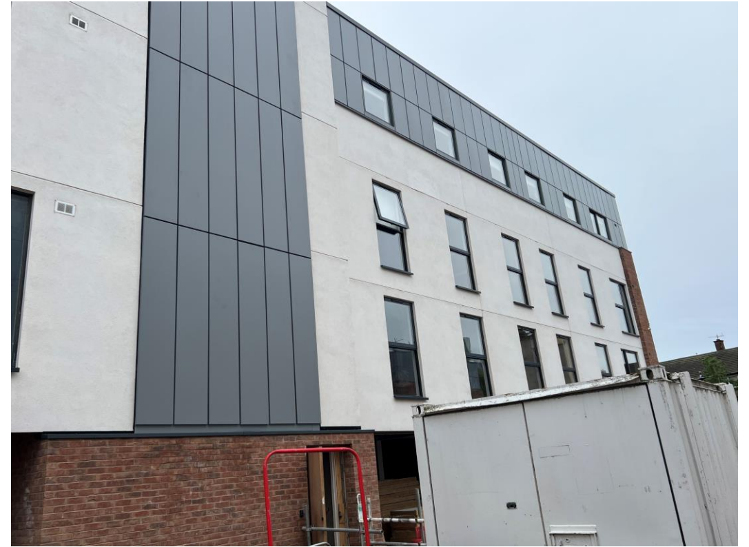
Residential Block – Cladding installation nearing completion
