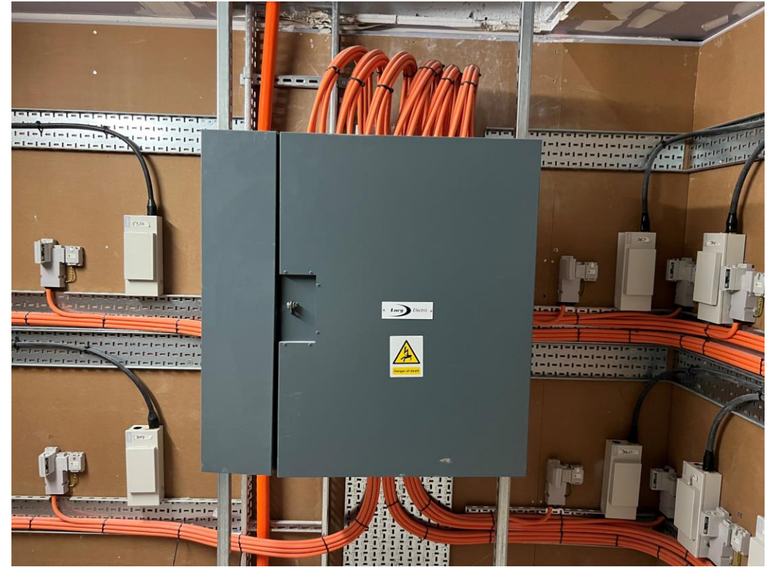
Residential Block – Apartment metres installation
