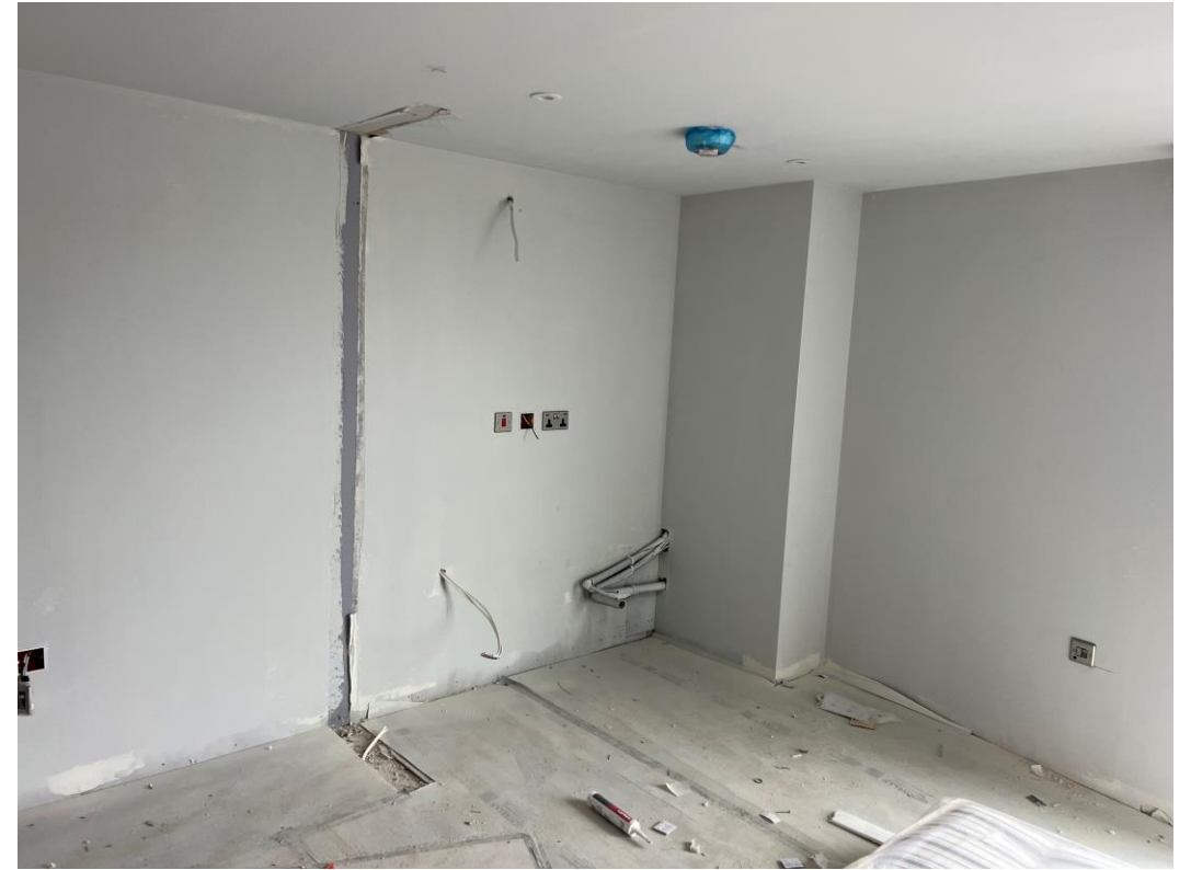
Residential Block – Decoration works on-going
