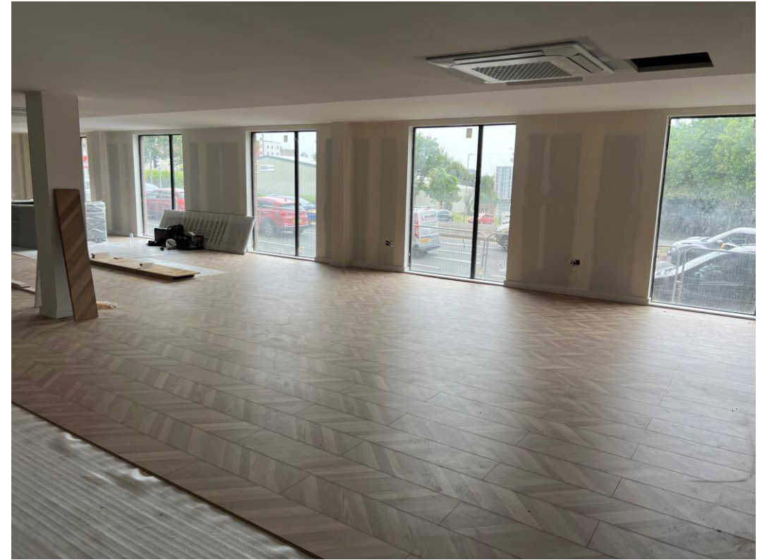
Ground Floor– Laminate flooring installation commenced
