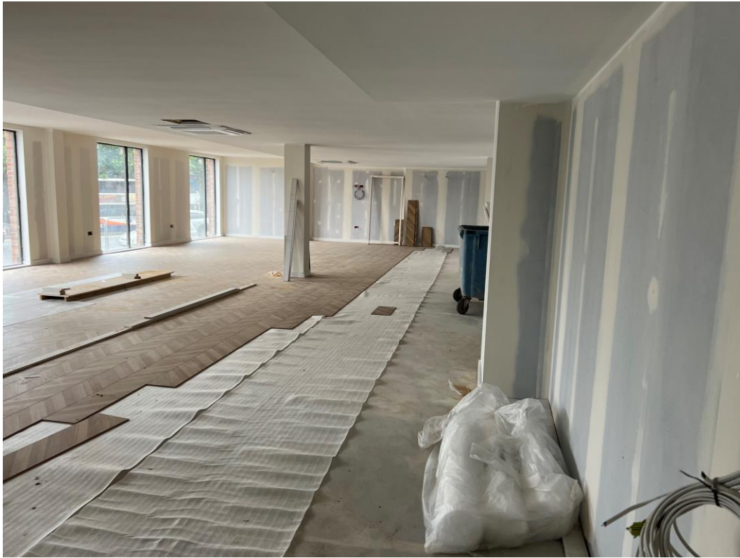
Ground Floor– Laminate flooring installation commenced
