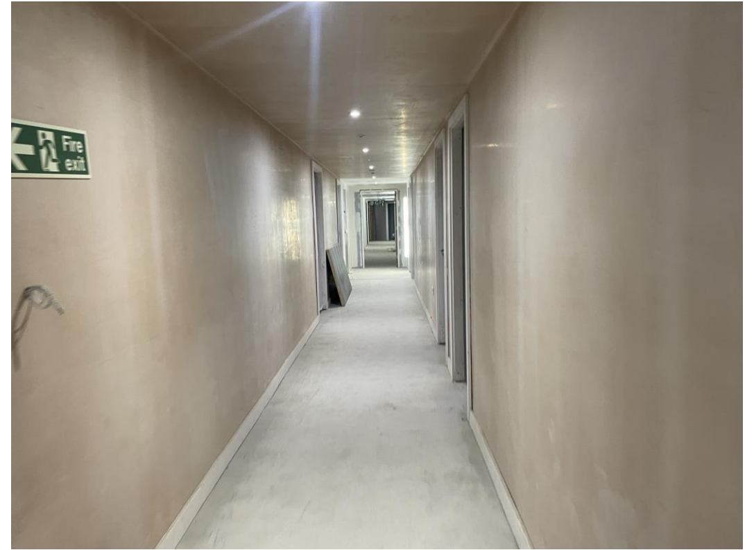
Student / Residential Wing – Latex screed applied
