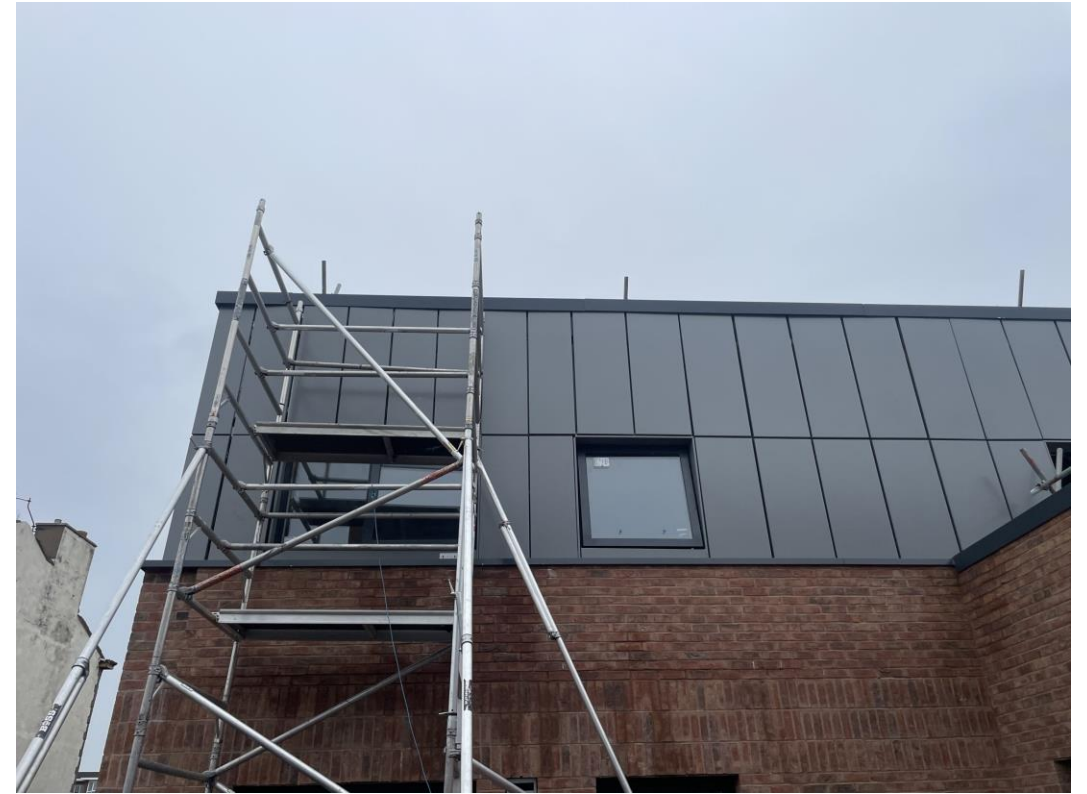
Commercial Units - Cladding installation nearing completion
