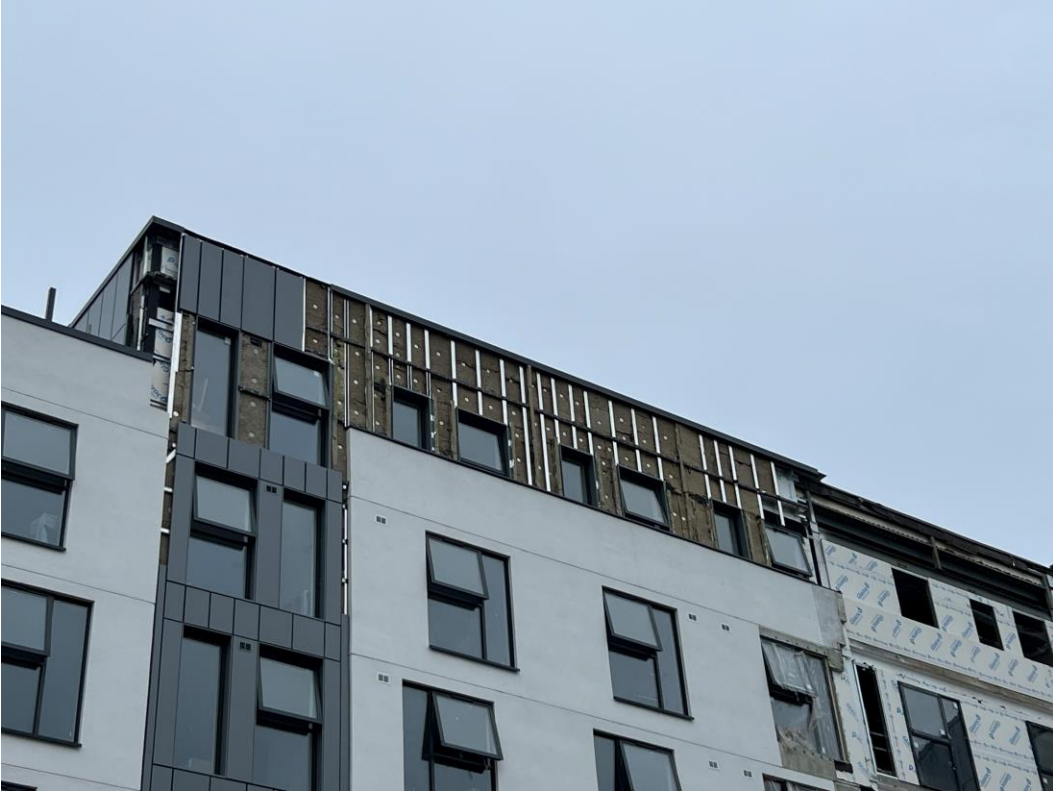
Student Wing – Cladding installation nearing completion
