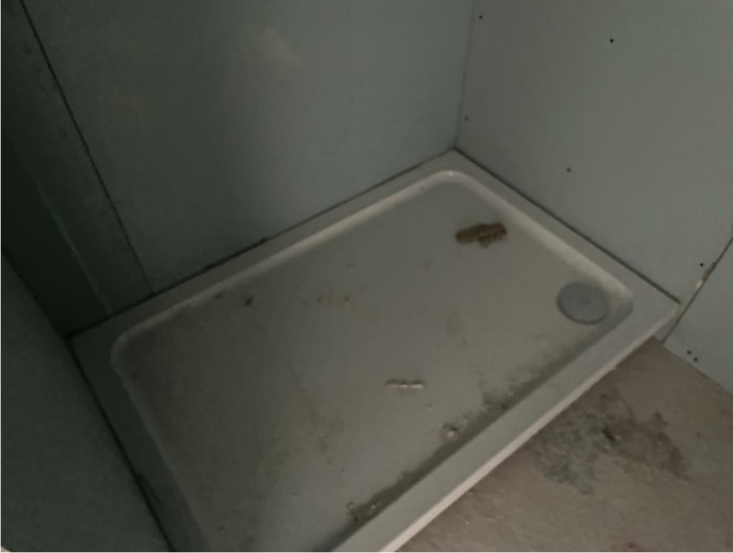
Residential Block – Shower tray installed
