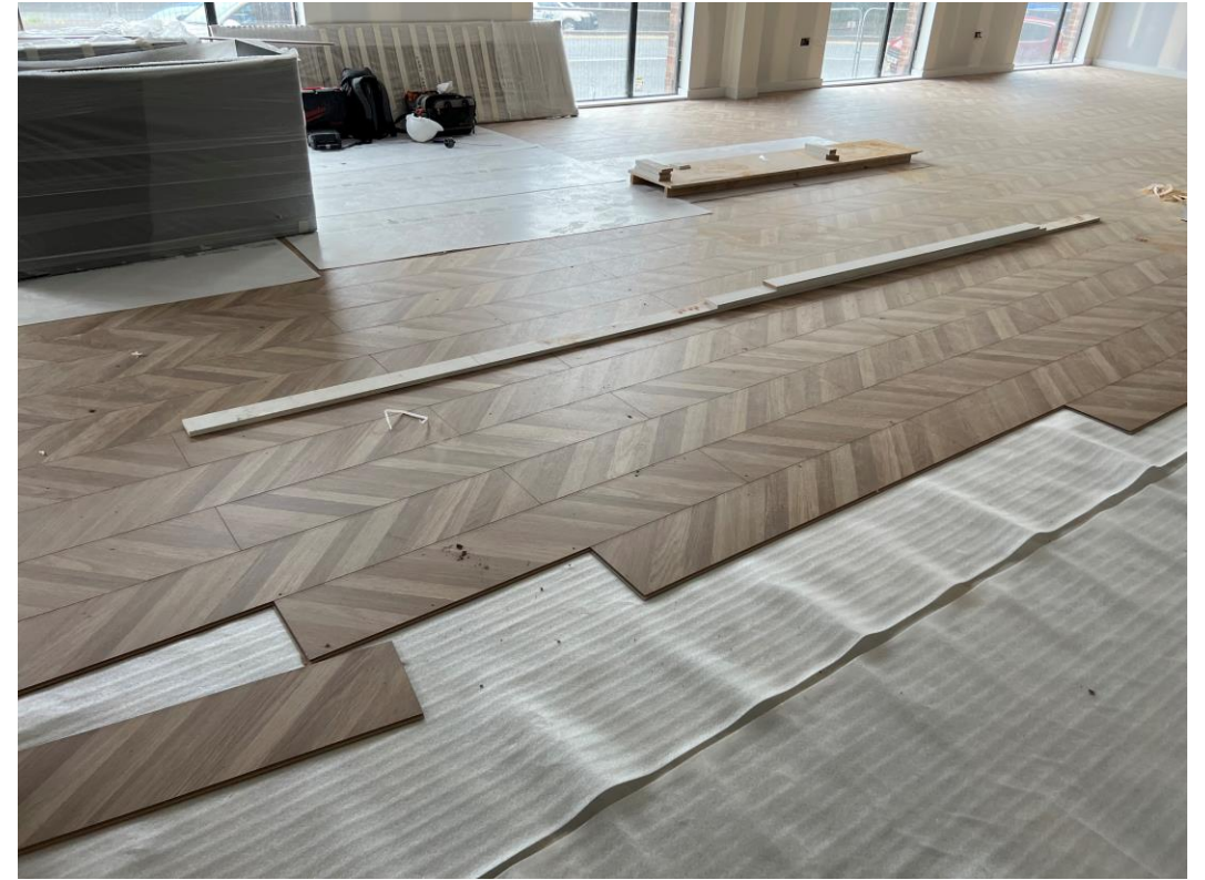
Ground Floor– Laminate flooring installation commenced
