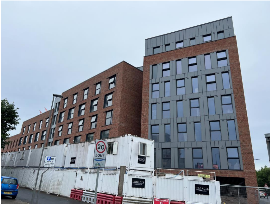
West Derby Road - Site view
