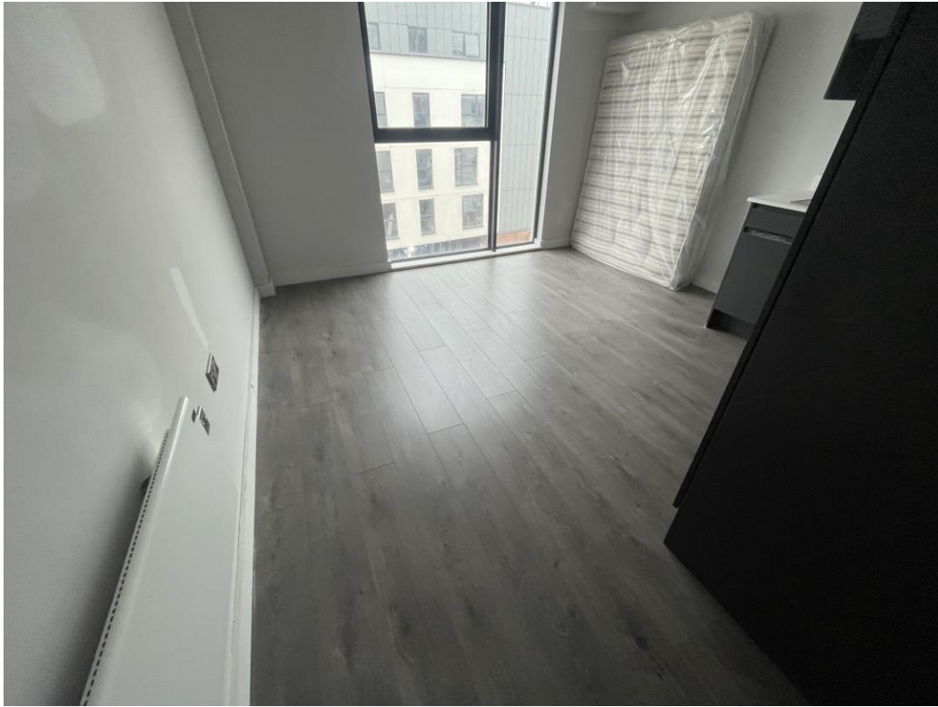
Residential Block – Laminate flooring installed
