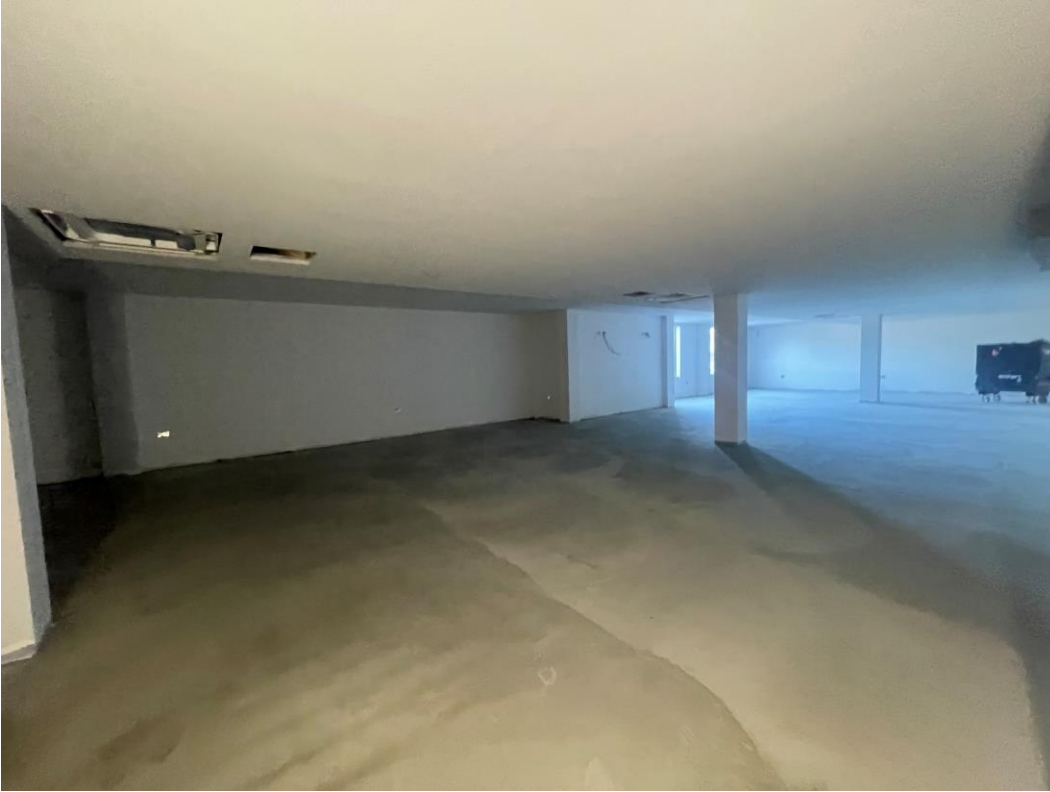
Ground Floor – Wall & ceiling decoration
