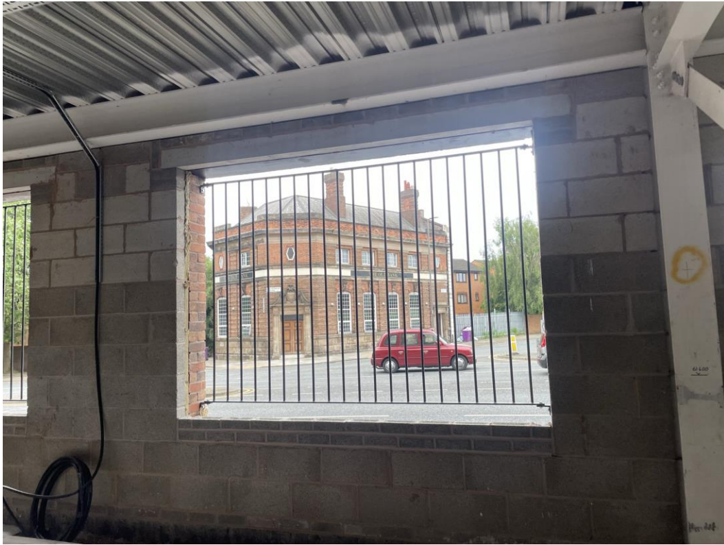
Under croft Car Park – Railings installed
