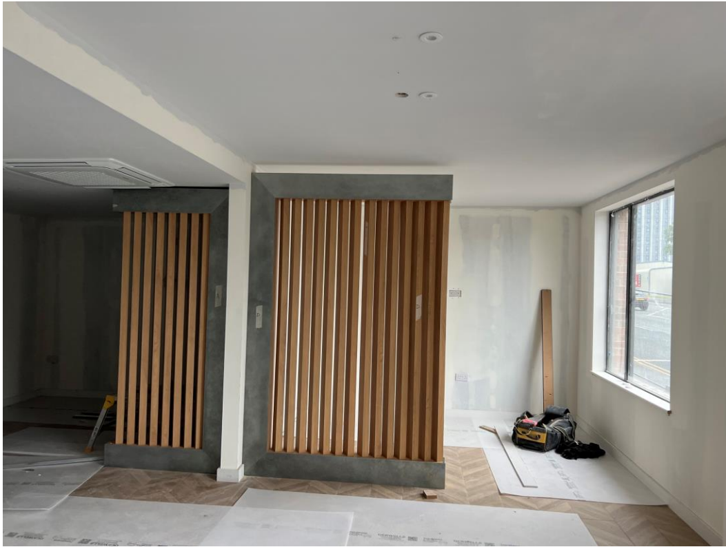
Ground Floor – Slattered Timber detail
