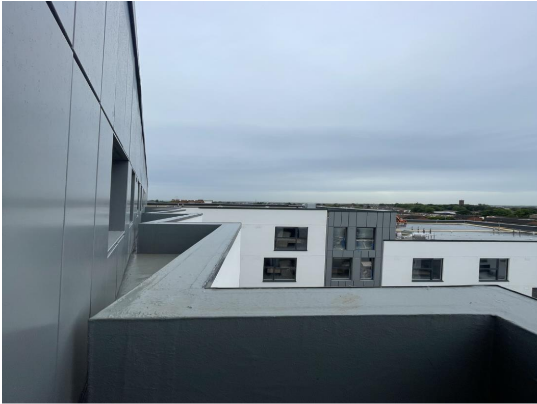
Liquid system applied to parapet walls
