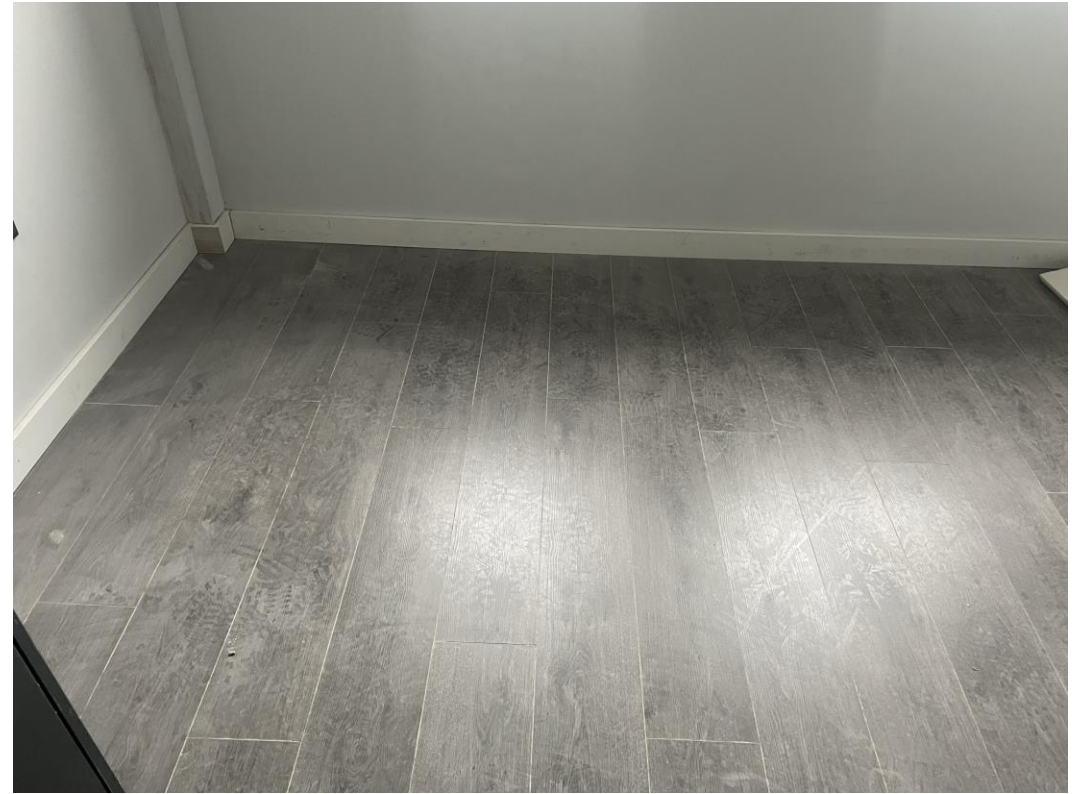
Residential Block – Laminate flooring installed
