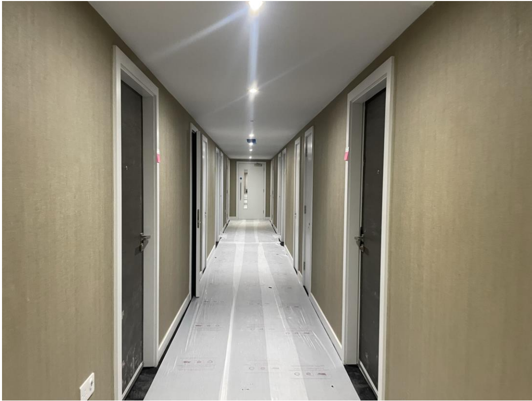
Student Block – Corridor Carpet tiles installed
