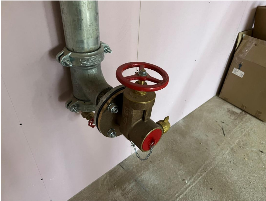
Residential Block – Dry Riser installation on-going
