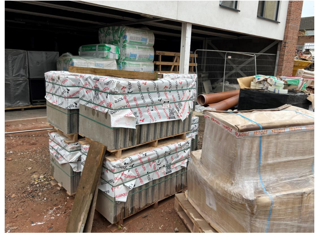
Material Storage – Paving slabs
