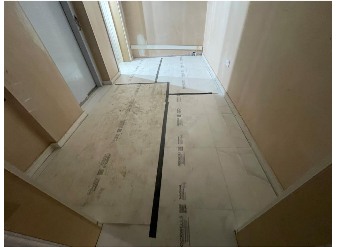
Student Block – Lift Lobby floor tiled
