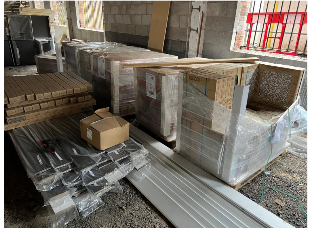
Material Storage – Ceramic floor tiles
