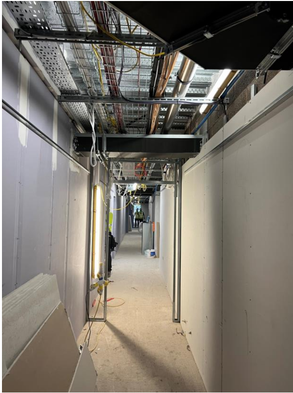
Ground Floor – Corridor walls boarded
