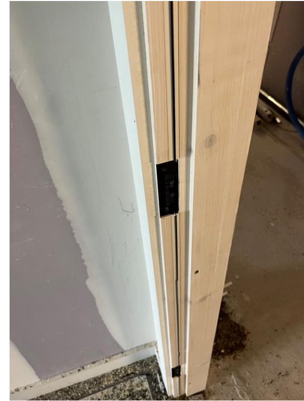
Residential Block – Apartment Door installation
