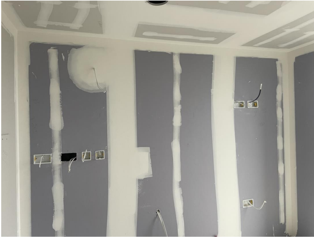
Residential Block – Walls & ceiling tape & jointed
