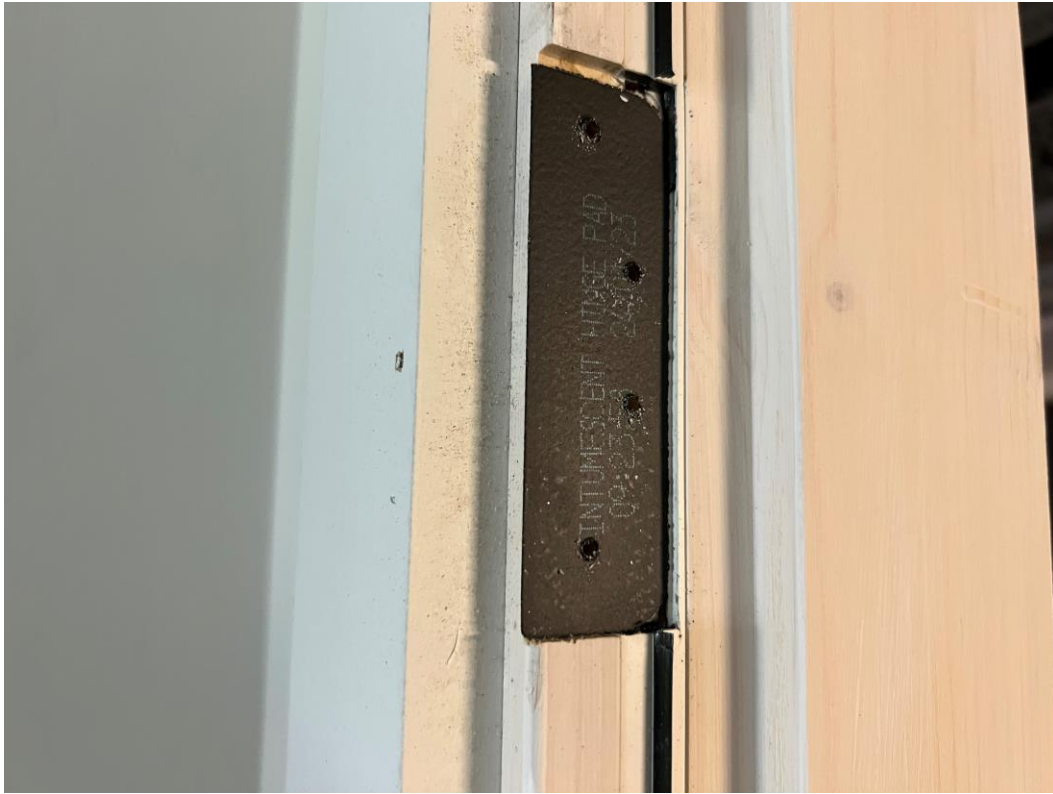
Residential Block – Apartment Door installation
