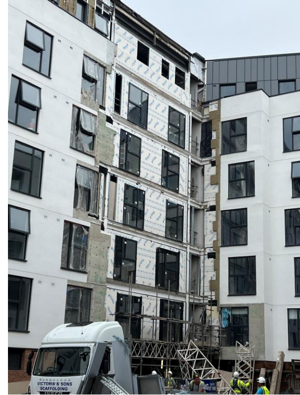
Residential Block – Removal of Hoist Lift
