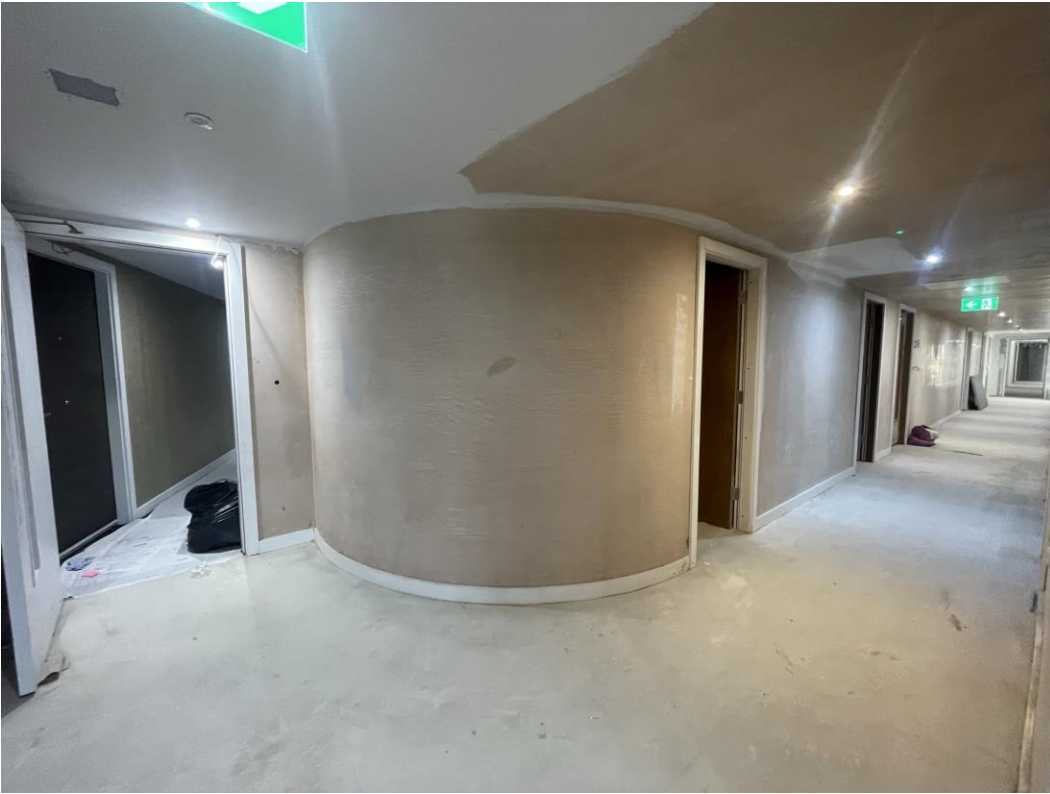
Residential Block – Walls & ceilings plastered
