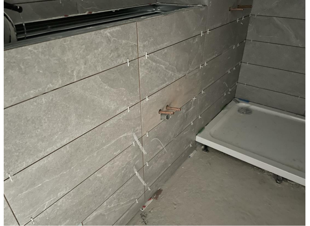
Residential Block – Wall tiles installed
