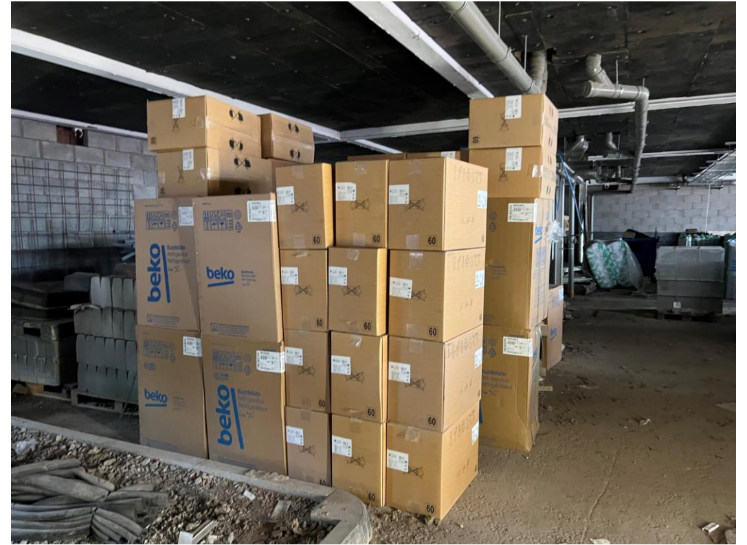
Material Storage – Sanitary Appliances
