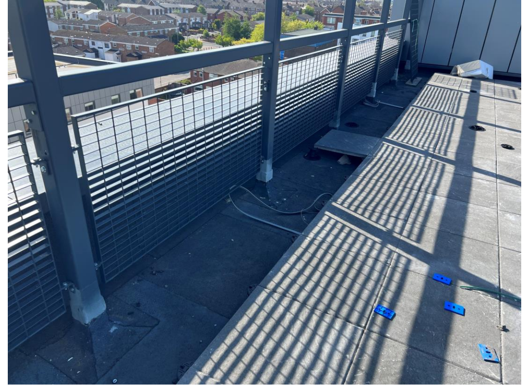
Residential Wing – Installation of metal balustrade commenced
