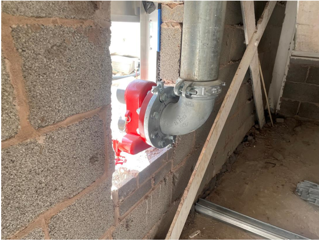
Residential Block – Dry Riser installation on-going
