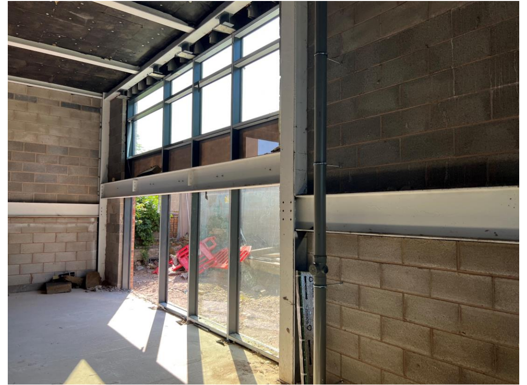
Commercial Block - Curtain walling
