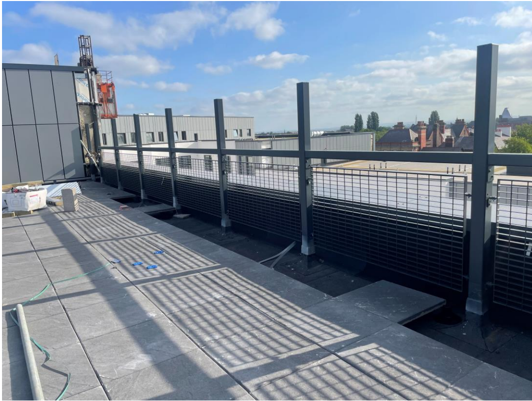
Residential Wing – Installation of metal balustrade commenced
