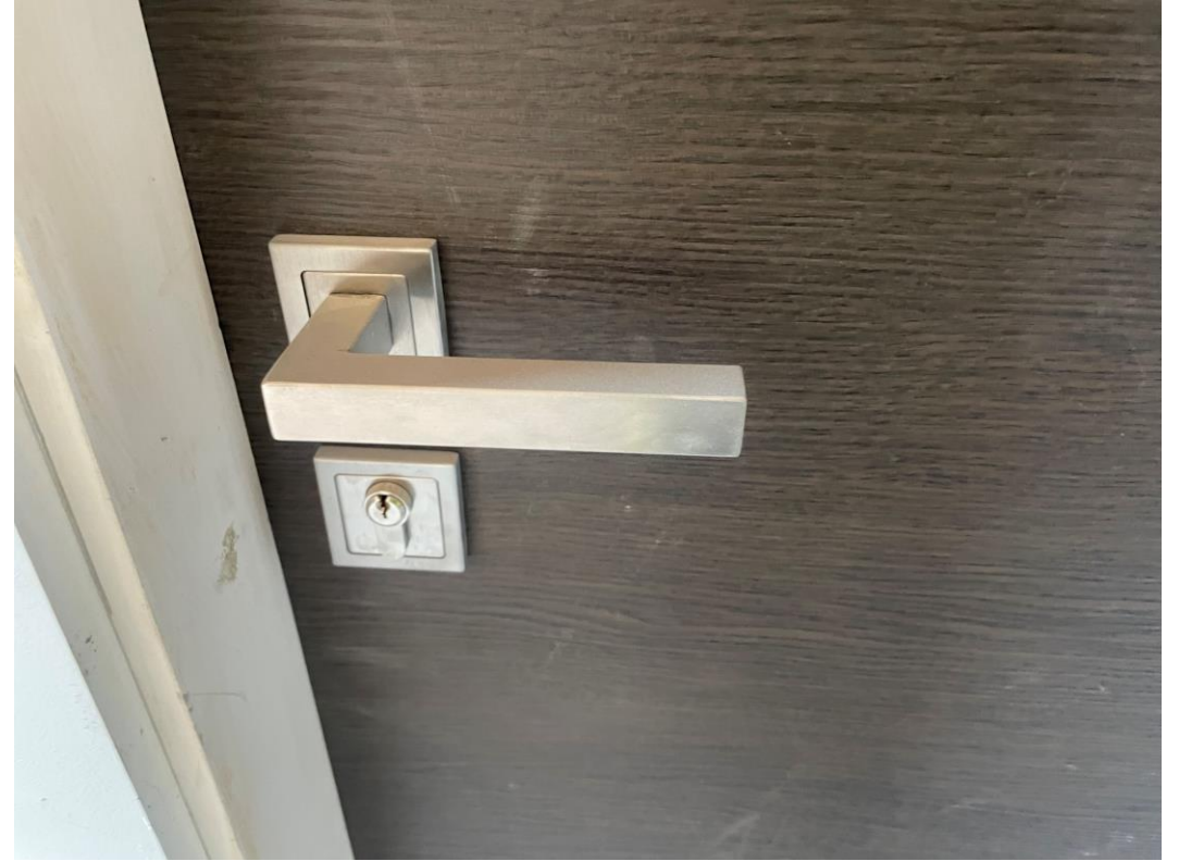
Residential Wing – Ironmongery installation
