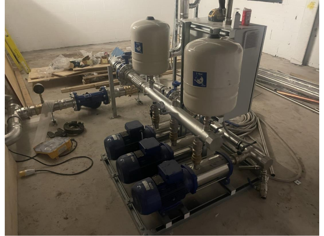
Residential Block – Water pump installation on-going
