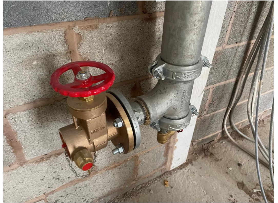
Residential Block – Dry Riser installation on-going
