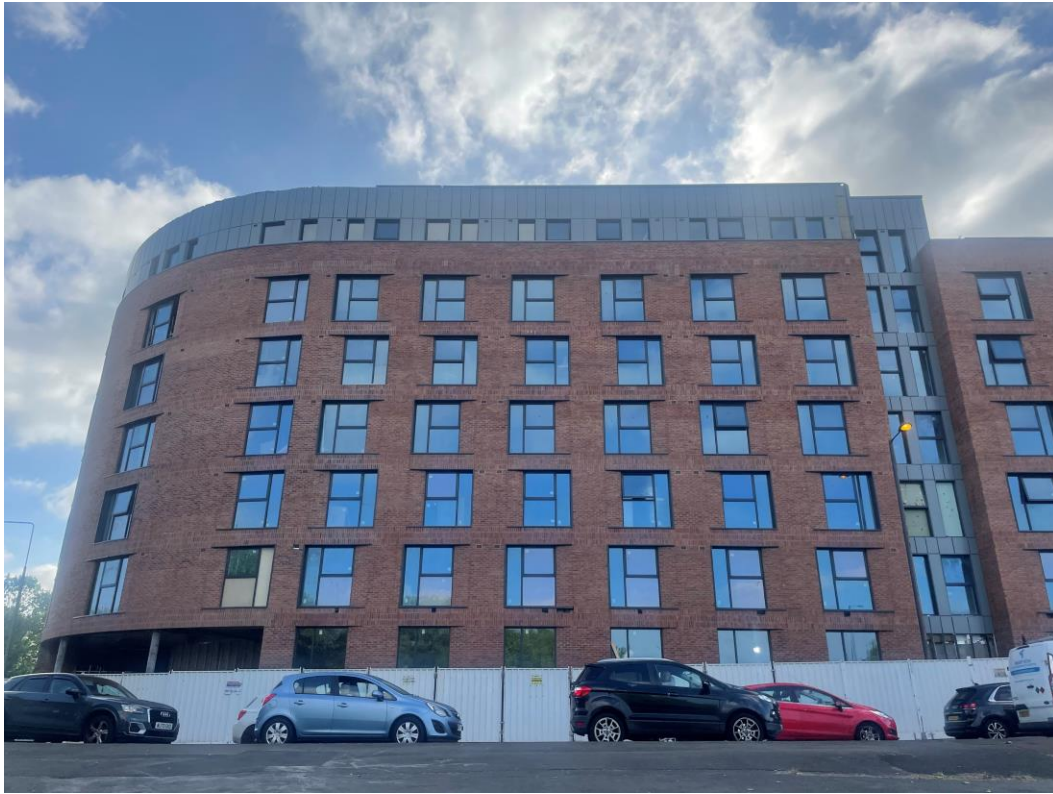
Brunswick Road - Site view
