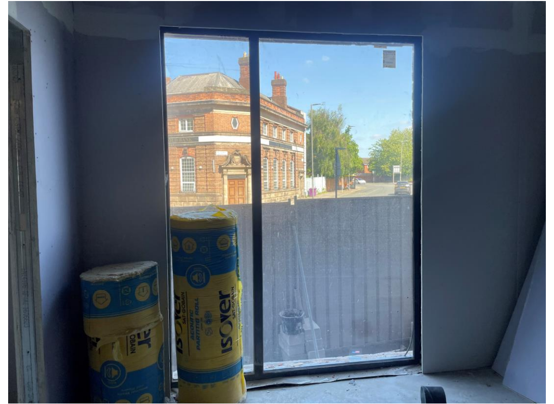
Residential Block – Boarding out of window wall
