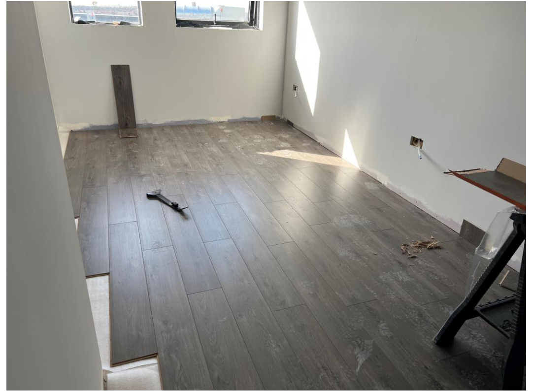
Residential Block – Laminate flooring installation on-going
