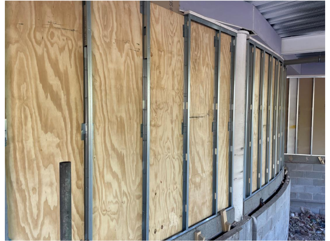
Residential Wing – Partitions erected & pattrass installed
