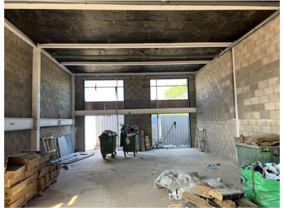
Commercial Block – Ceiling soffit insulation detail installed
