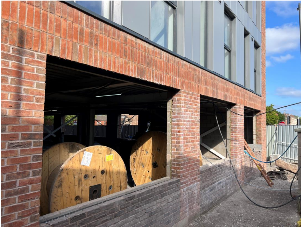
Commercial Block – Scaffolding removal complete
