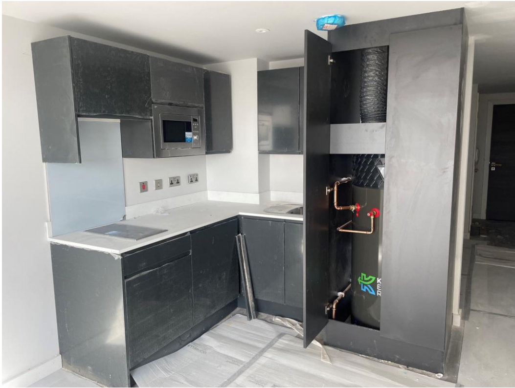
Residential Wing – Kitchen installation
