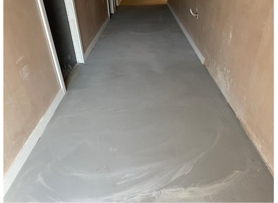
Student / Residential Wing – Latex screed applied
