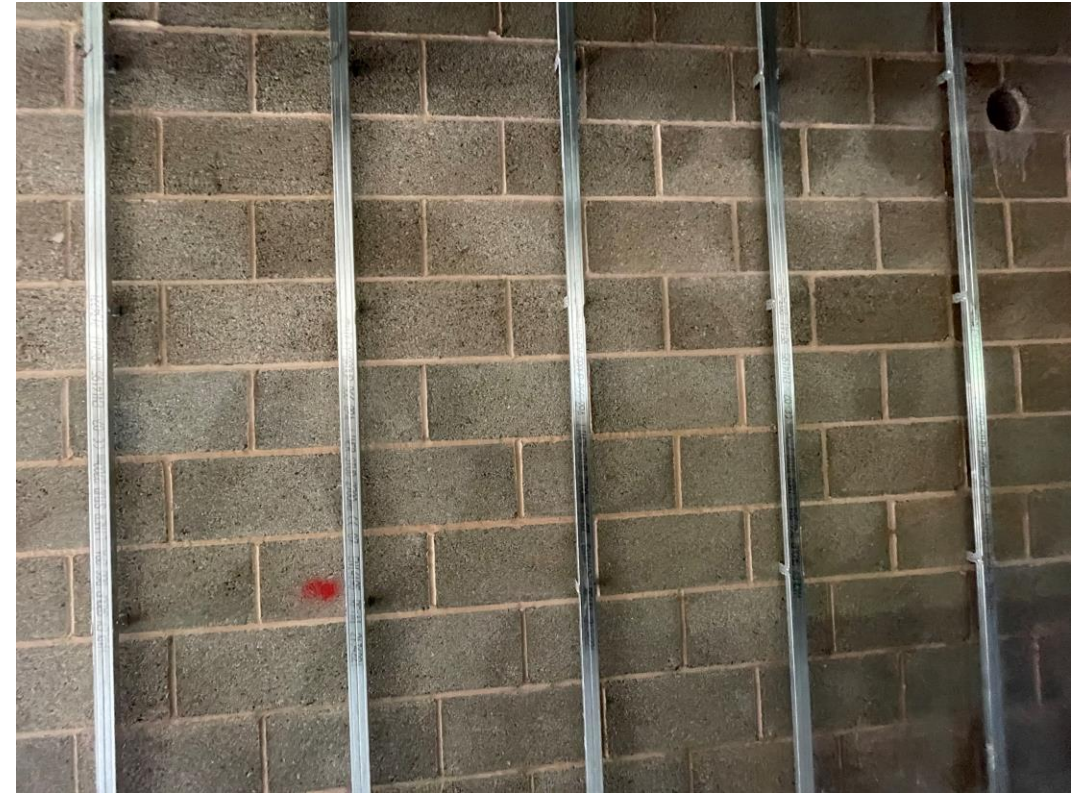
Residential Block – Metal partitions erected
