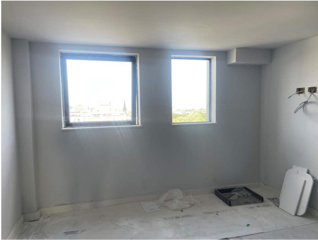
Residential Block – Decoration works on-going
