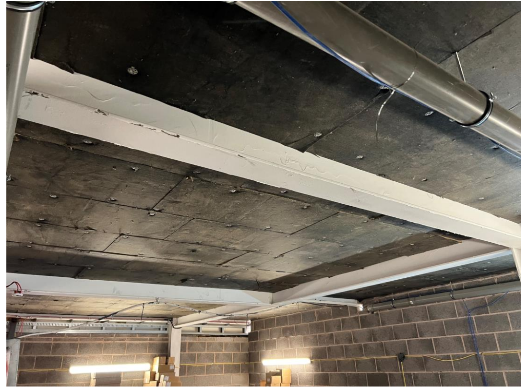
Residential Block – Ceiling soffit insulation installed
