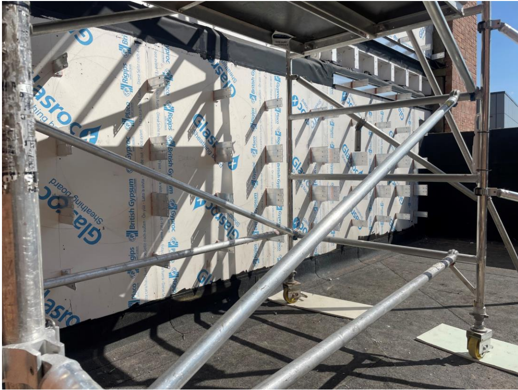
Rainscreen cladding rails installation on-going
