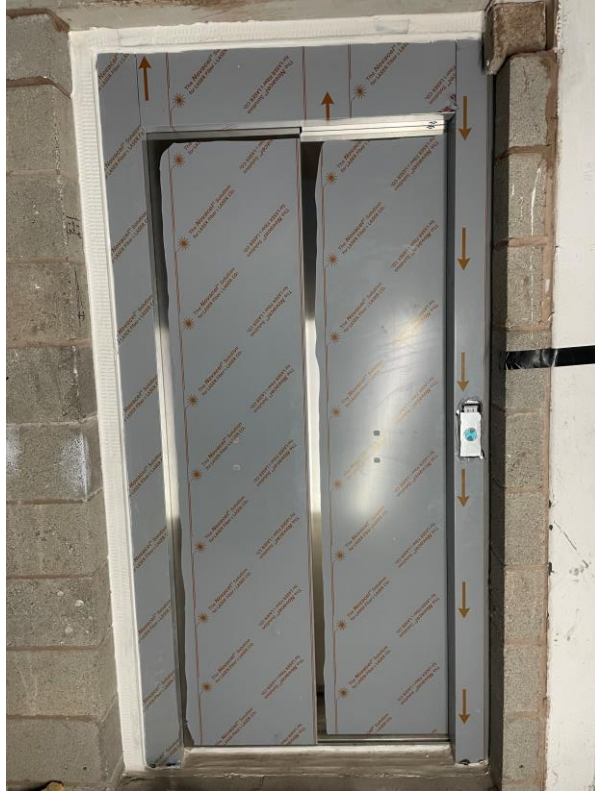
Student Block – Fire stopping to lift surround complete
