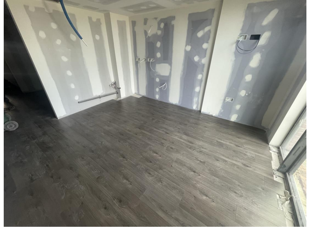
Residential Block – Laminate flooring installed
