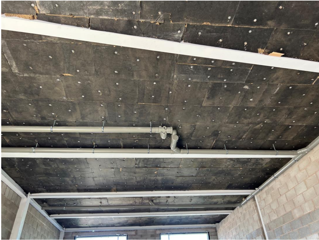
Commercial Block – Ceiling soffit insulation detail installed
