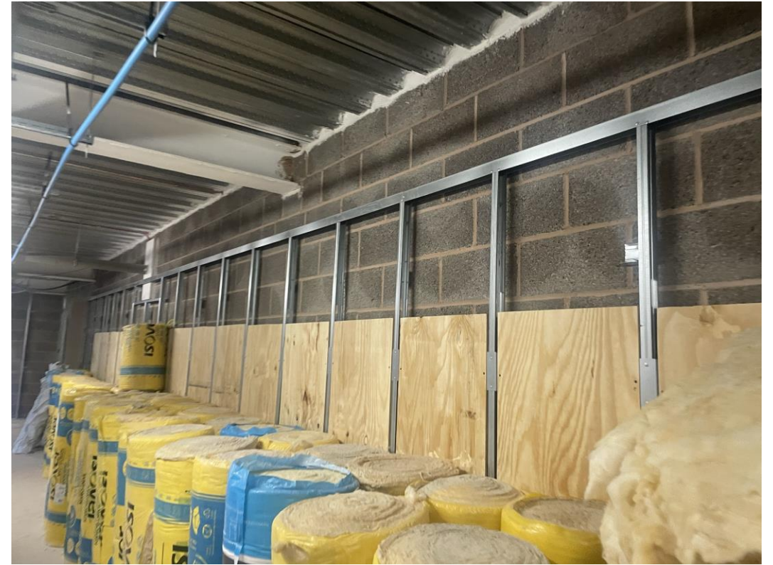
Material Storage – Insulation
