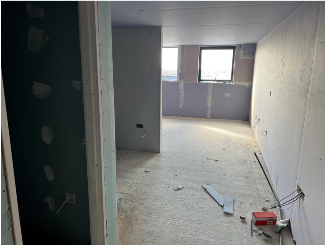
Residential Block – Walls & ceiling boarded
