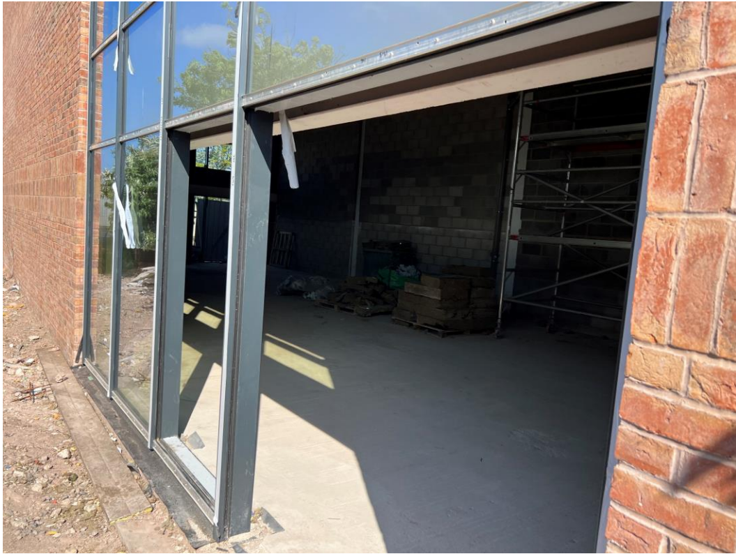
Commercial Block - Curtain walling
