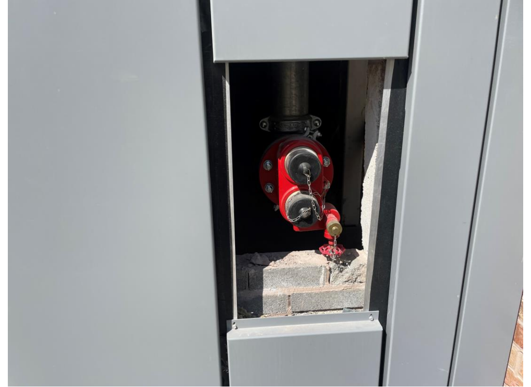
Dry riser installation on-going
