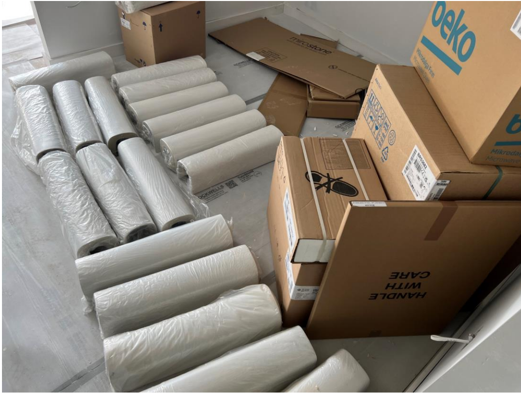
Material Storage – Sanitary Appliances
