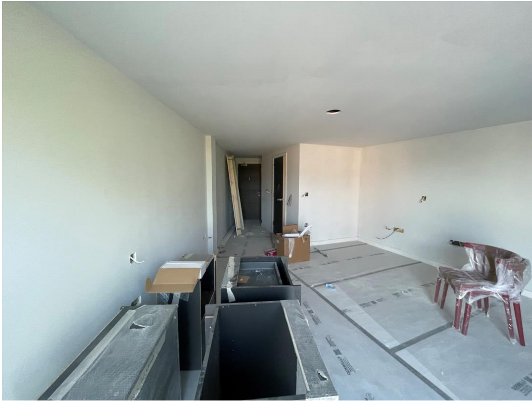
Residential Block – Decoration works on-going
