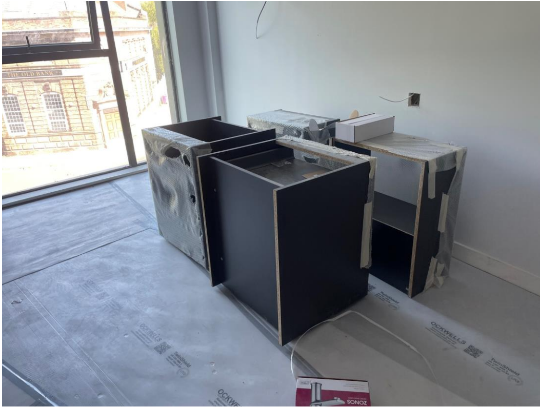
Material storage – Kitchen units
