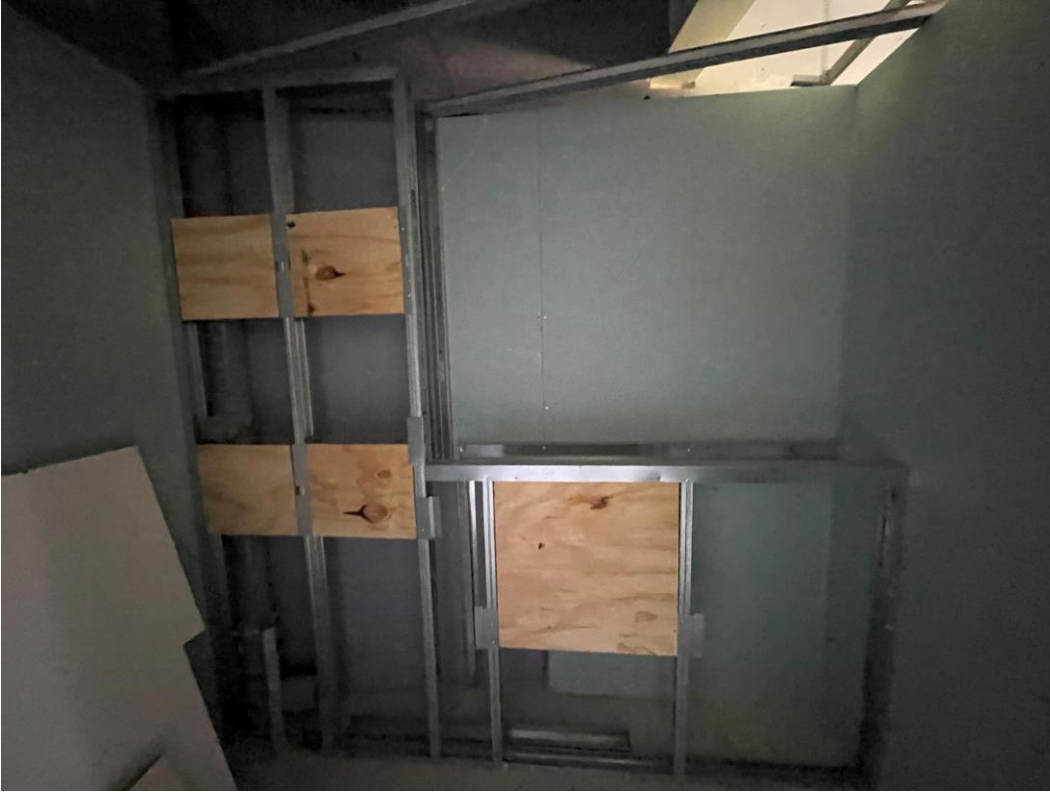
Residential Block – IPS Installed
