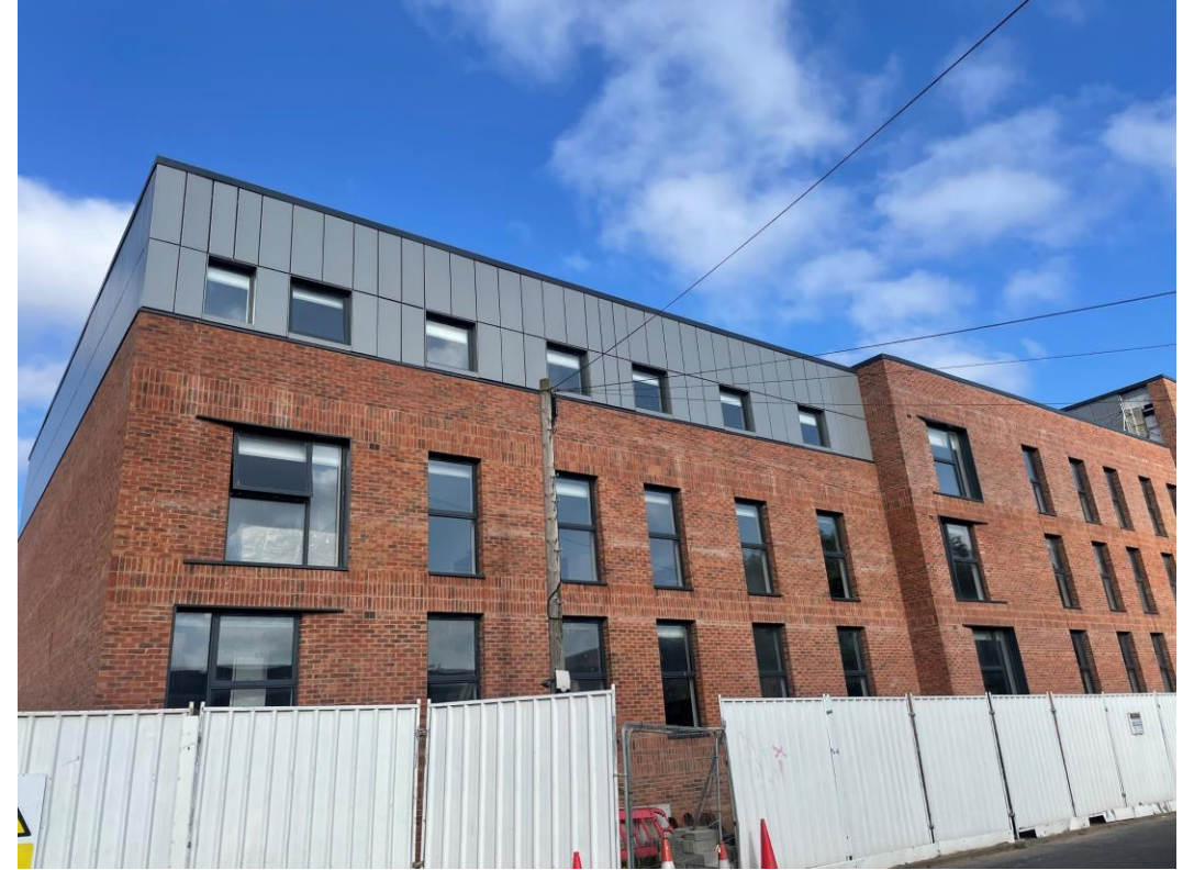
Walker Street - Site view
