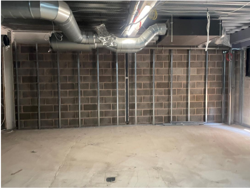
Residential Block – Metal partitions erected
