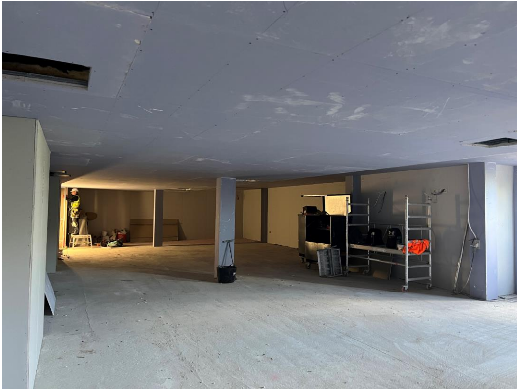
Residential Block – Ceiling insulated & boarded
