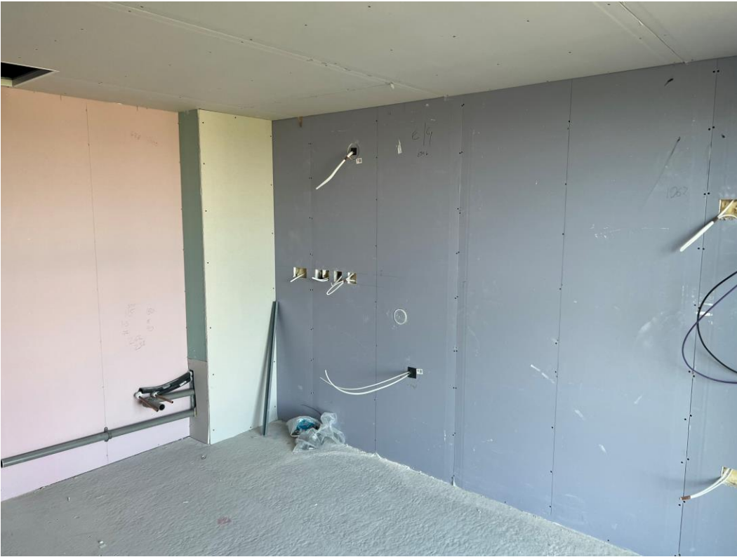
Residential Block – Walls & ceiling boarded
