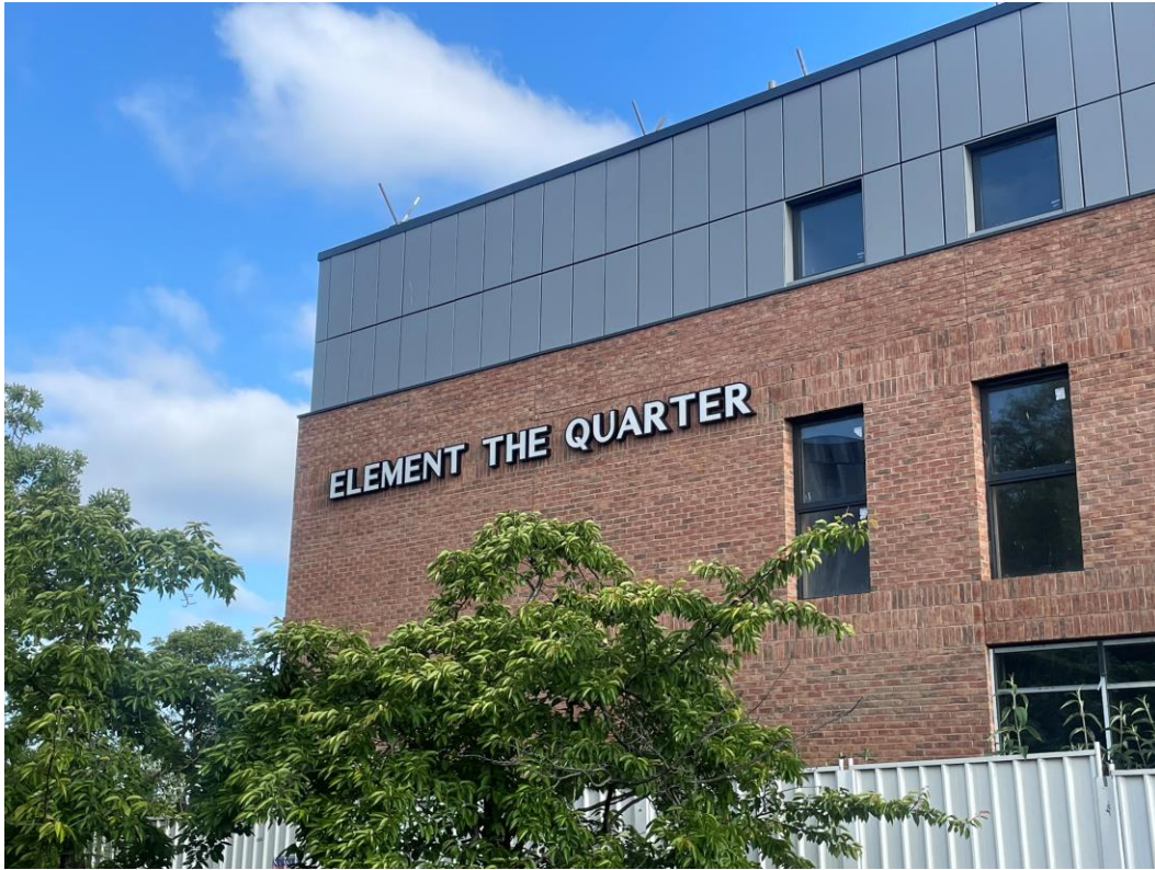
Brunswick Road –Building signage
