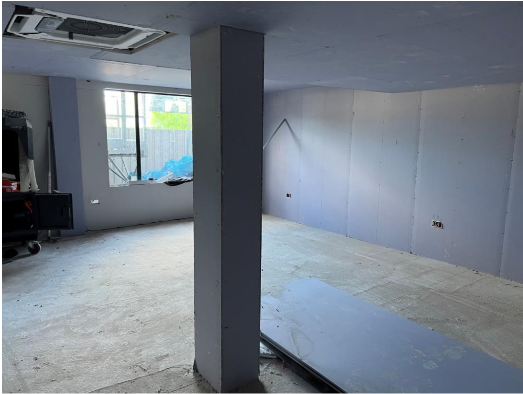
Ground Floor – Partitions boarded both sides
