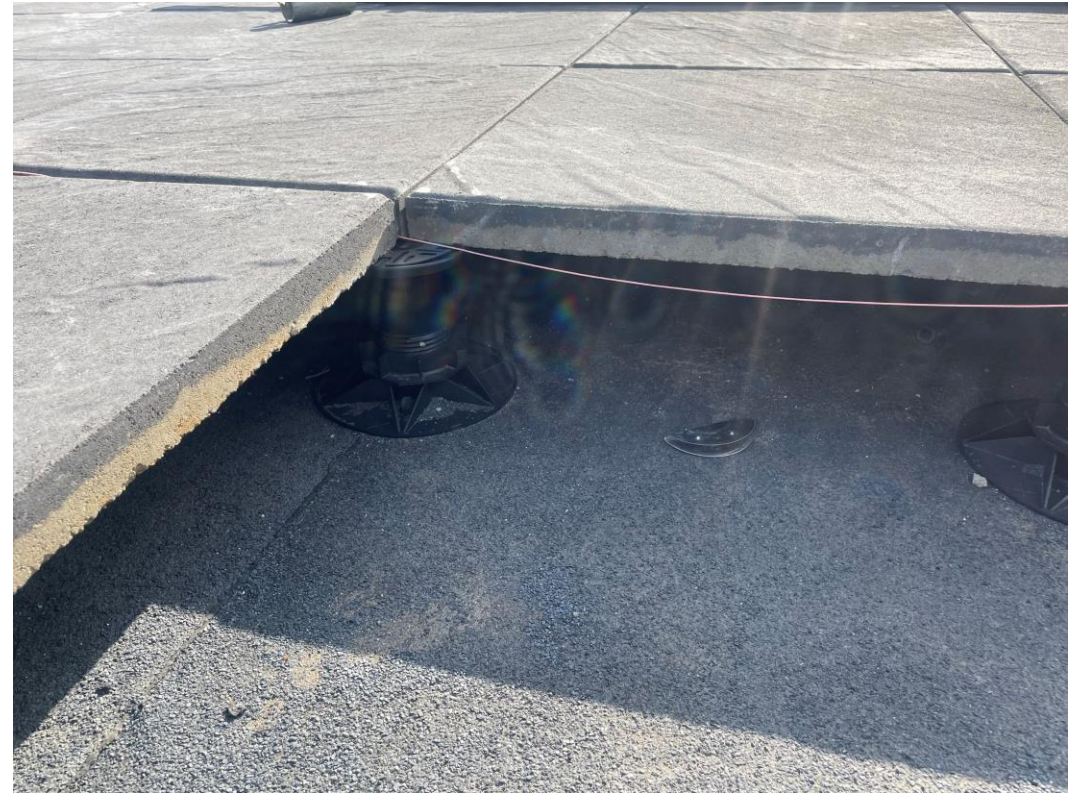
Residential Wing – Paving installation on-going
