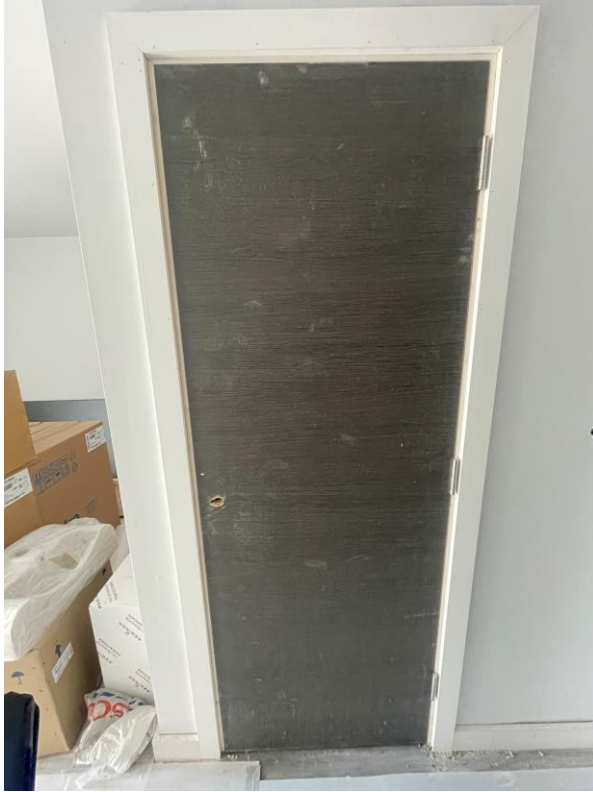
Residential Wing – Apartment doors installed
