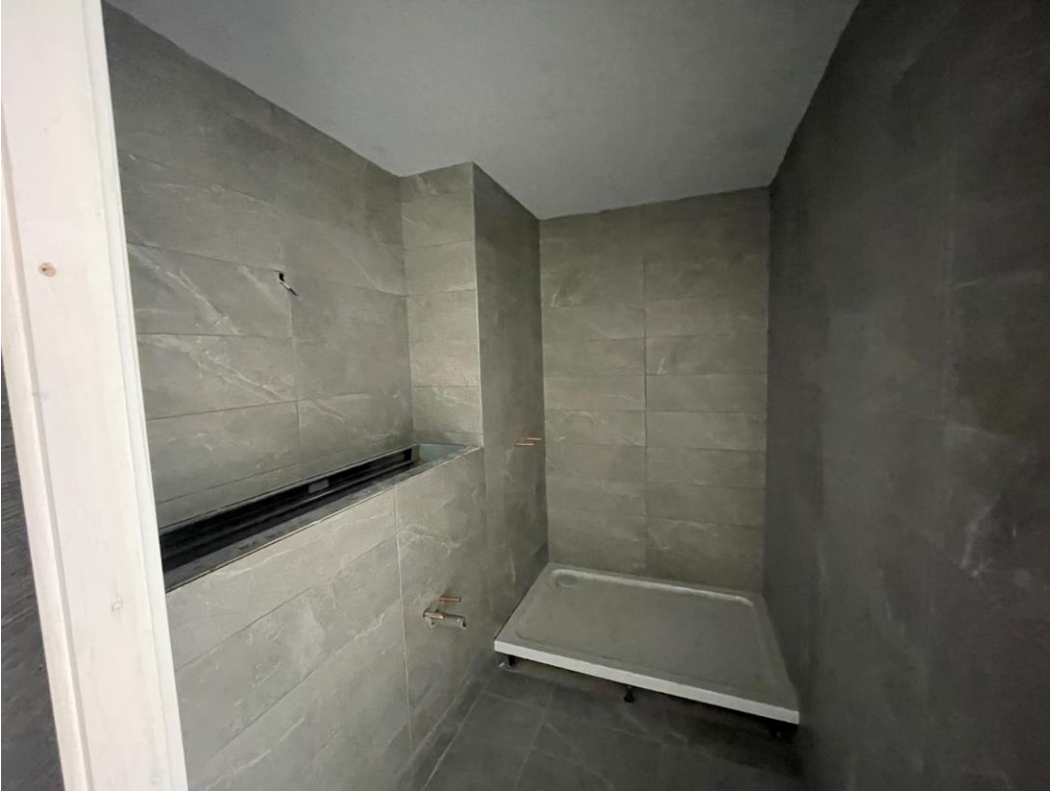
Residential Block – Floor & wall tiles installed
