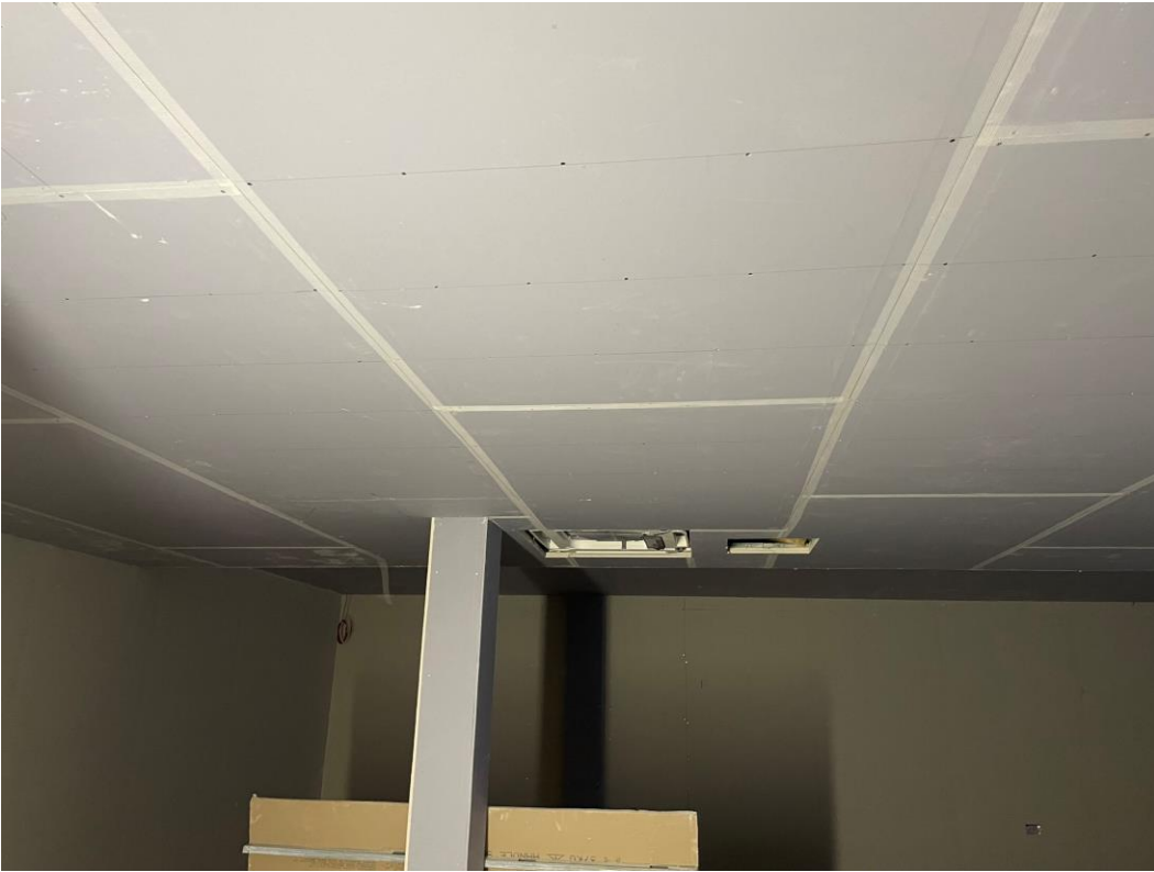
Residential Block – Ceiling insulated & boarded
