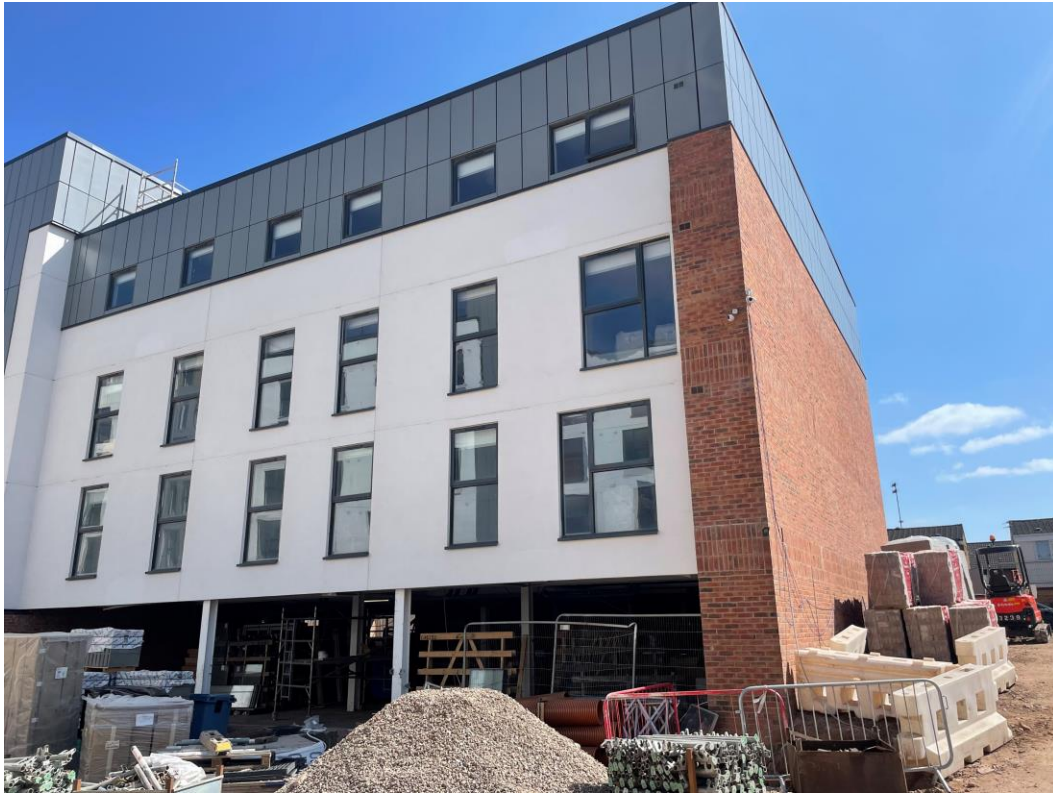
Student Wing – Cladding installation nearing completion
