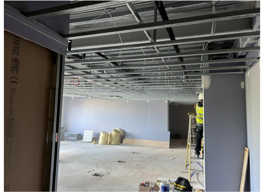
Residential Block – Metal ceiling grid erected
