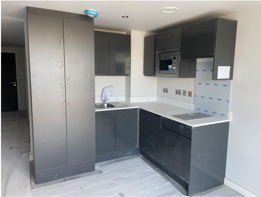
Residential Block – Kitchen complete
