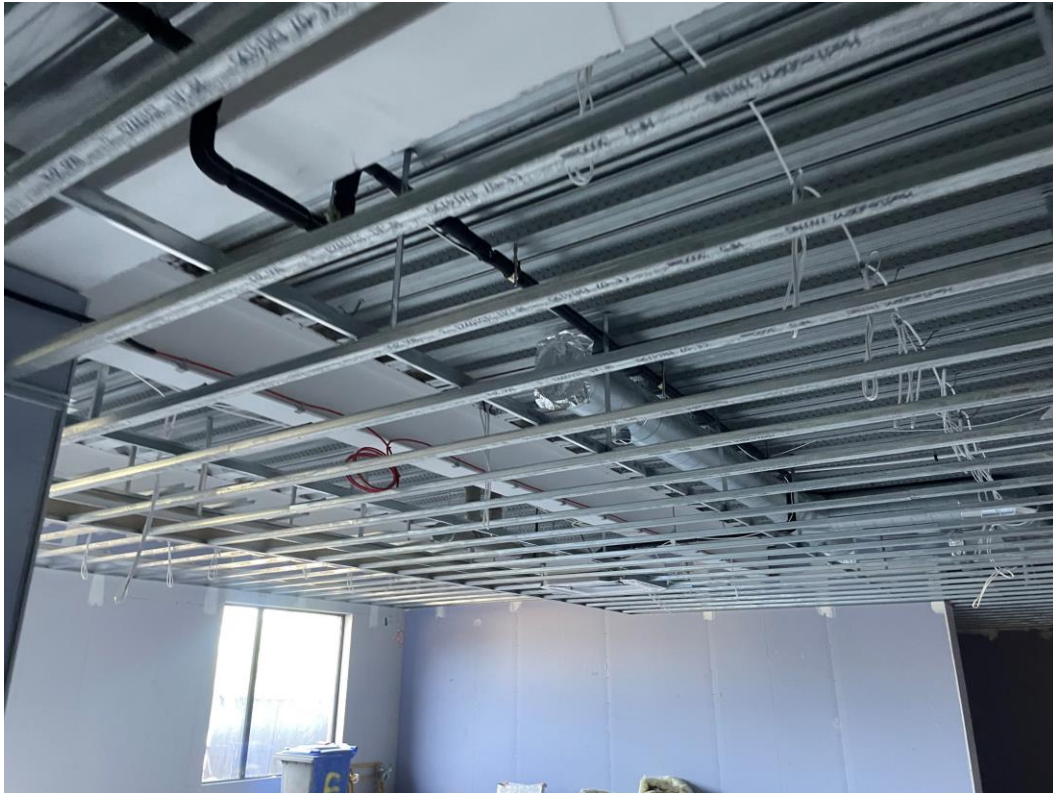
Residential Block – Metal ceiling grid erected
