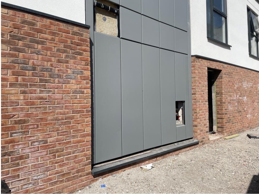
Commercial Units – Cladding nearing completion
