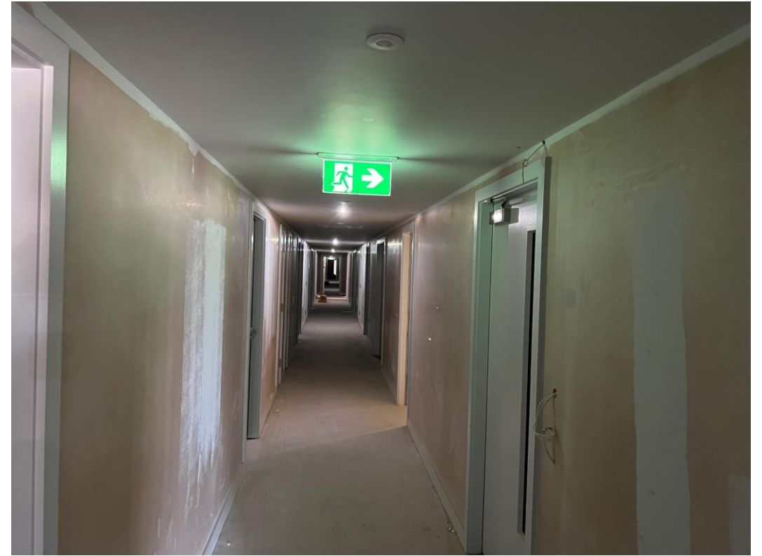
Student Wing – Way finding installed
