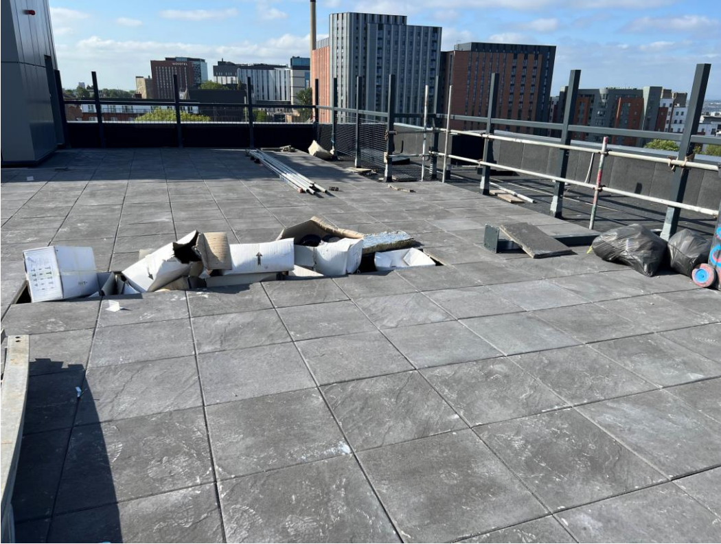
Residential Wing – Paving installation on-going
