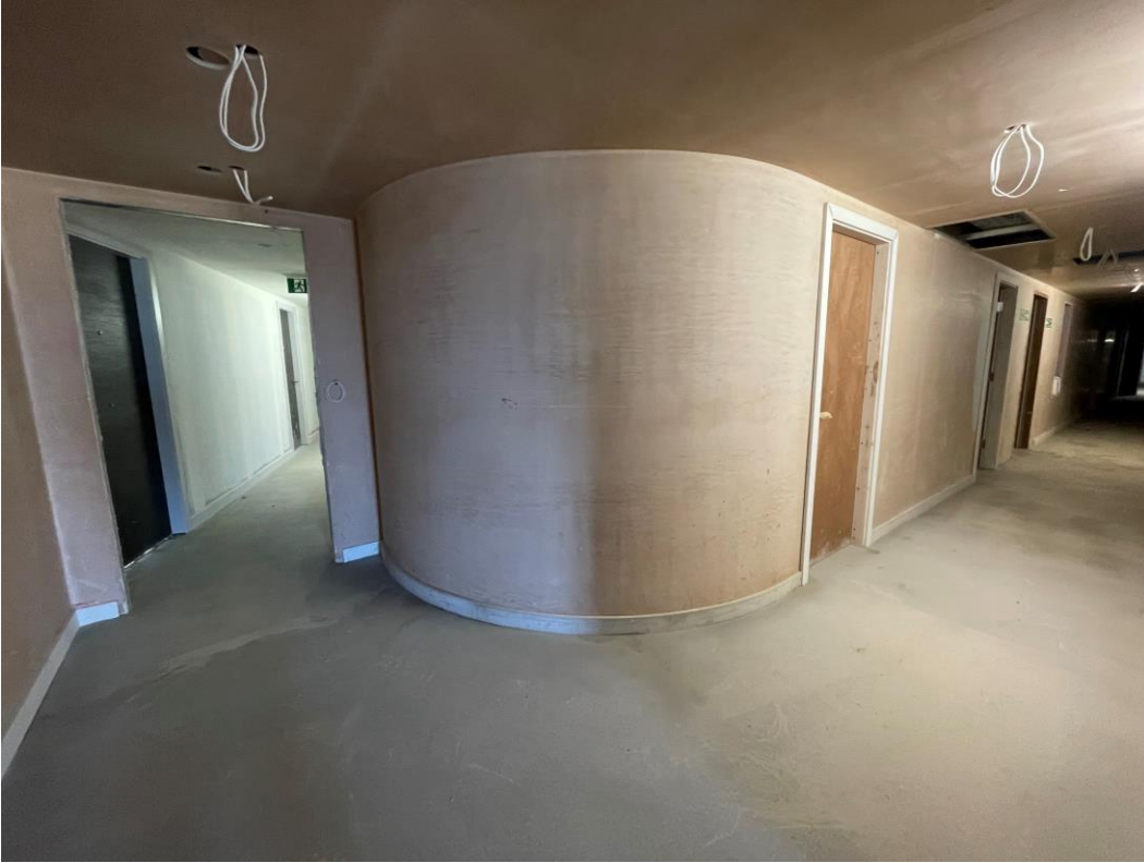
Residential Block – Walls & ceilings plastered
