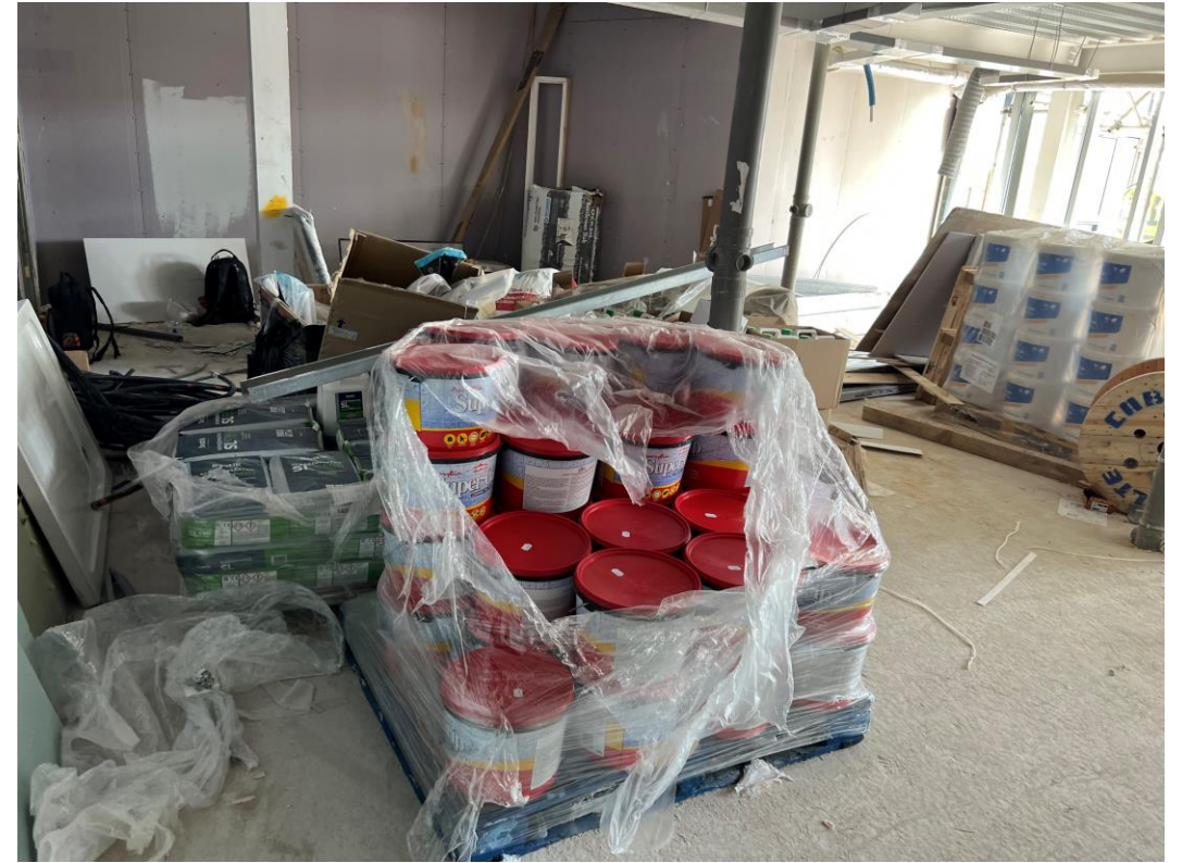
Material Storage – Tile Adhesive
