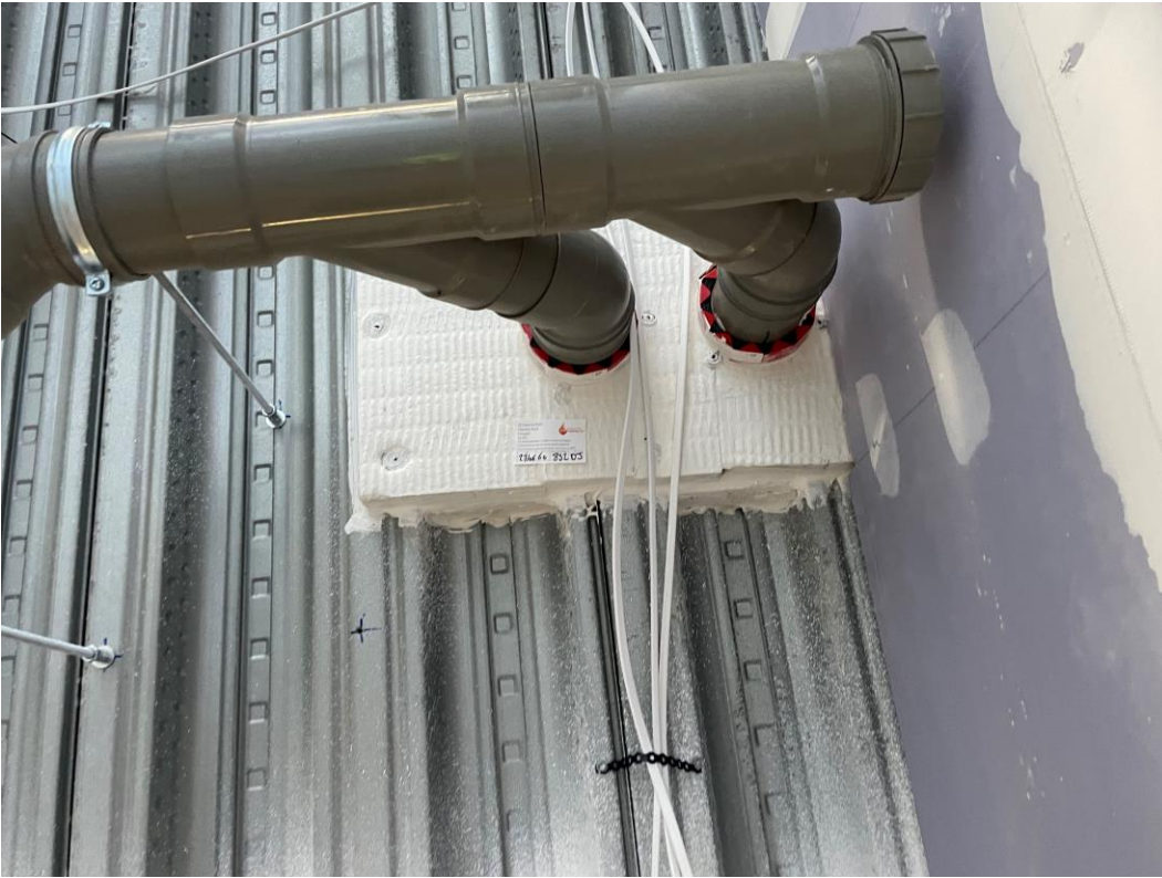
Fire stopping works
