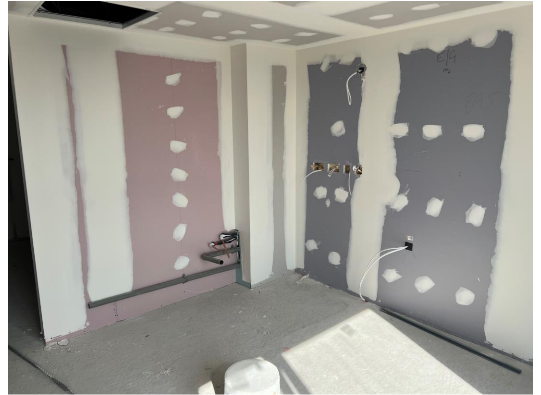
Residential Block – Tape & jointing on-going
