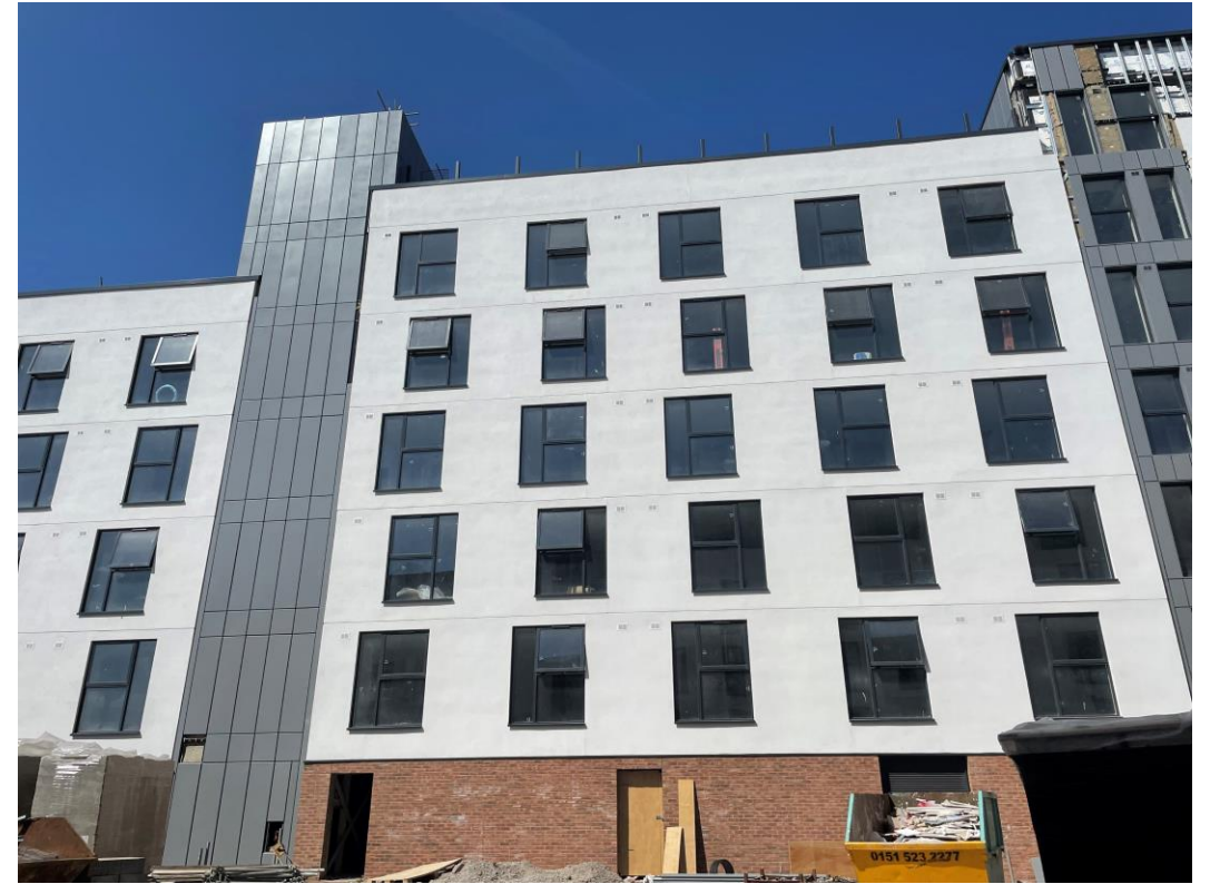
Residential Block – Cladding installation nearing completion
