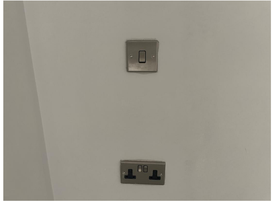
Residential Block – Light switches & sockets installed
