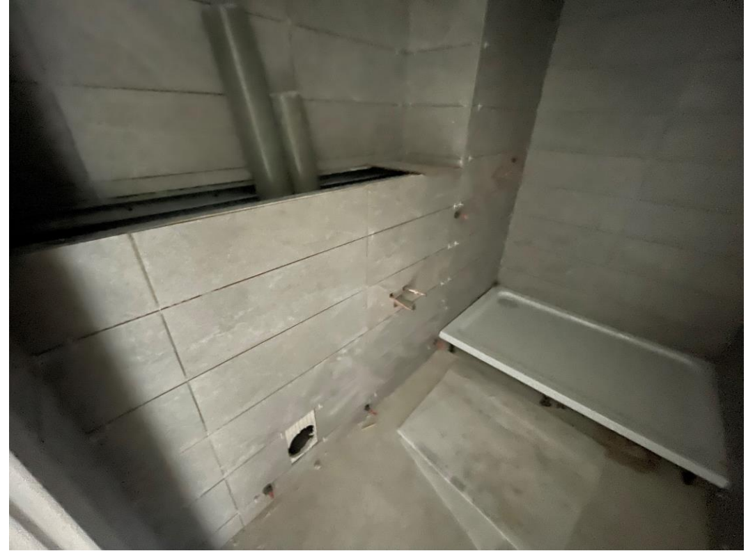
Residential Block – Wall tiles installed
