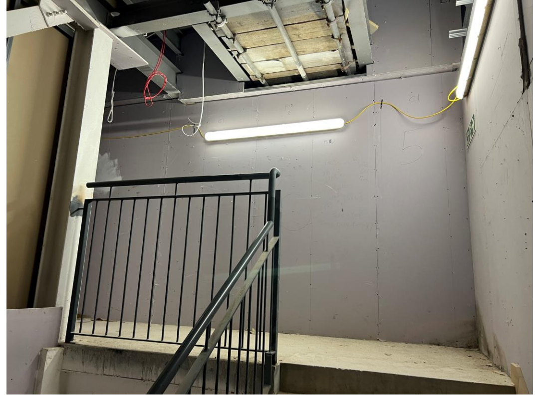
Student Block – Stairwell walls boarded
