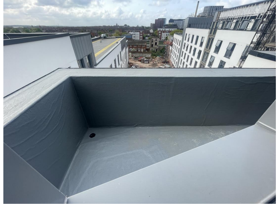
Liquid system applied to parapet walls
