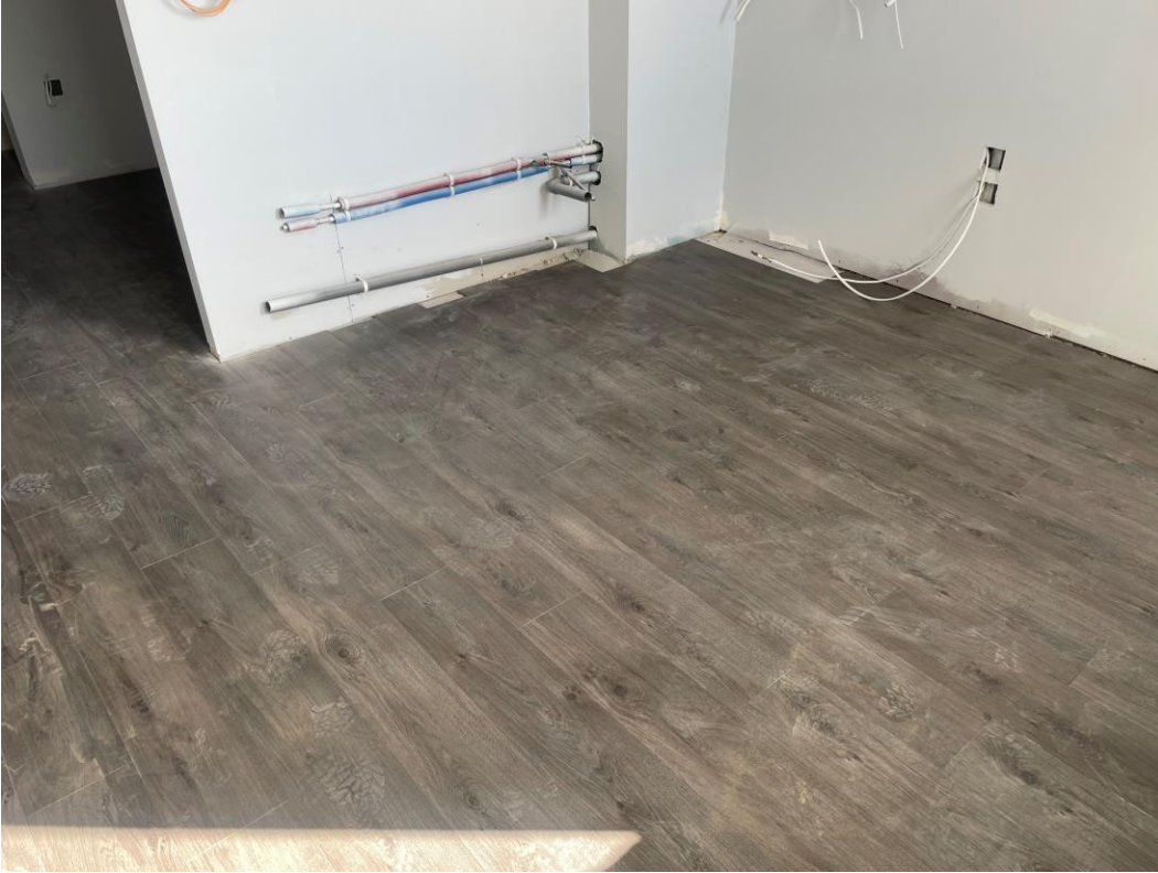
Residential Block – Laminate flooring installed
