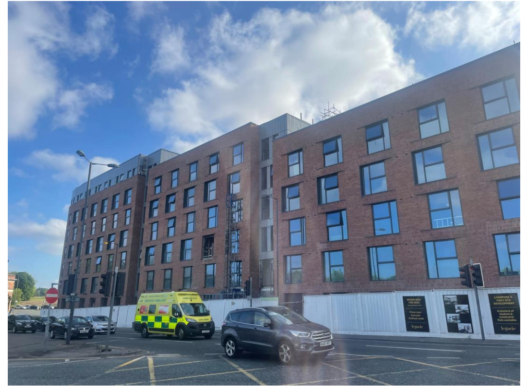
Brunswick Road - Site view
