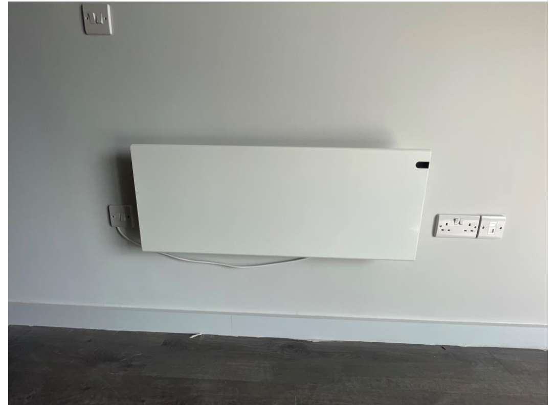
Residential Block – Radiator installation
