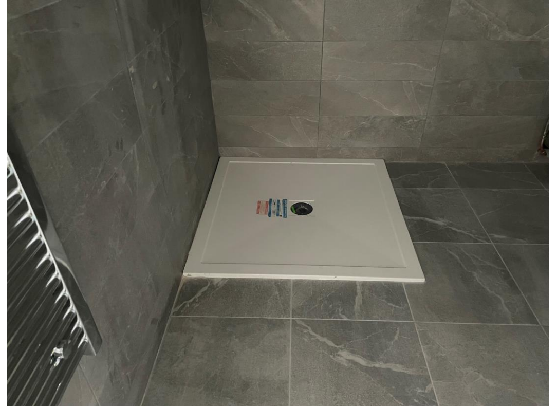
Residential Block – Shower tray installed
