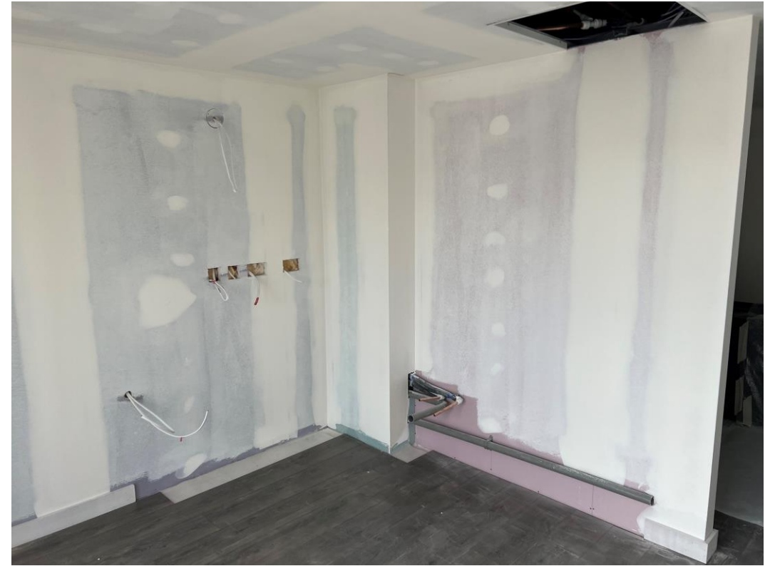
Residential Block – Mist coat applied to walls & ceilings
