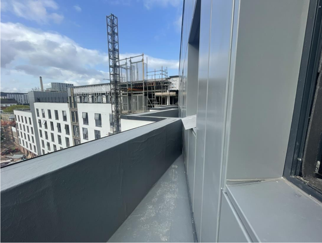
Residential Wing – Cladding installation nearing completion
