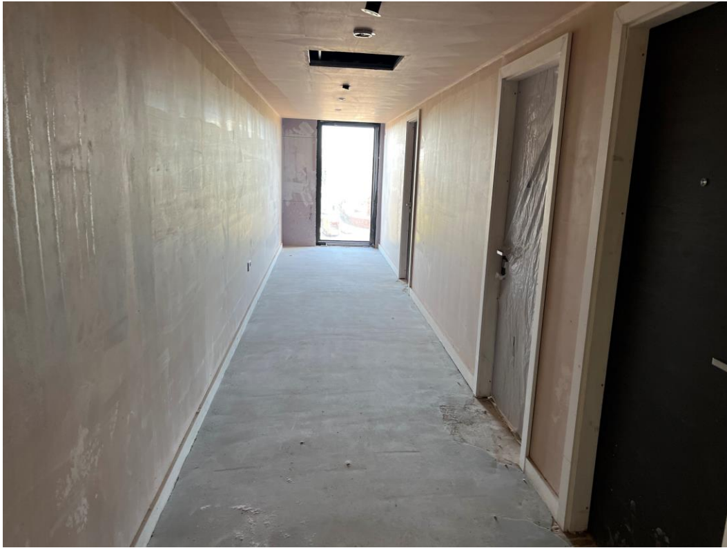
Residential Block – Corridor walls & ceiling plastered
