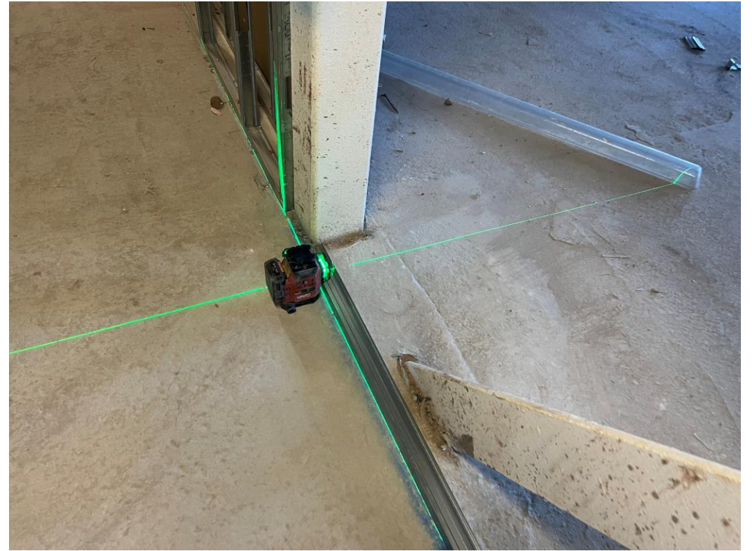
Residential Block – Setting out of partitions on-going
