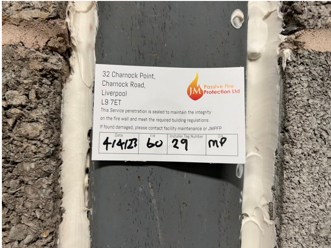
Fire stopping works
