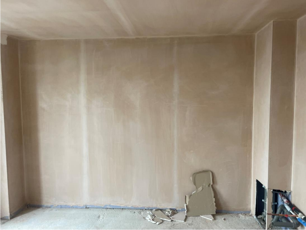
Residential Block – Walls & ceiling plastered
