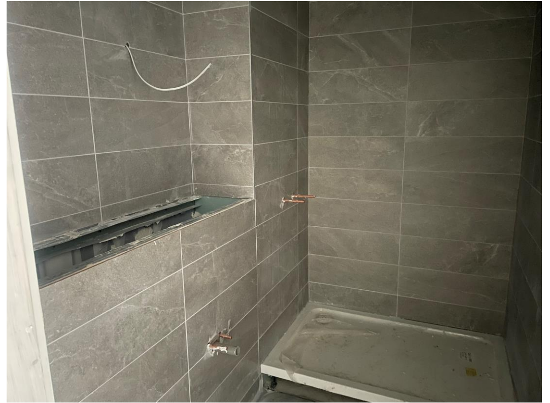
Residential Block – Wall tiles installed
