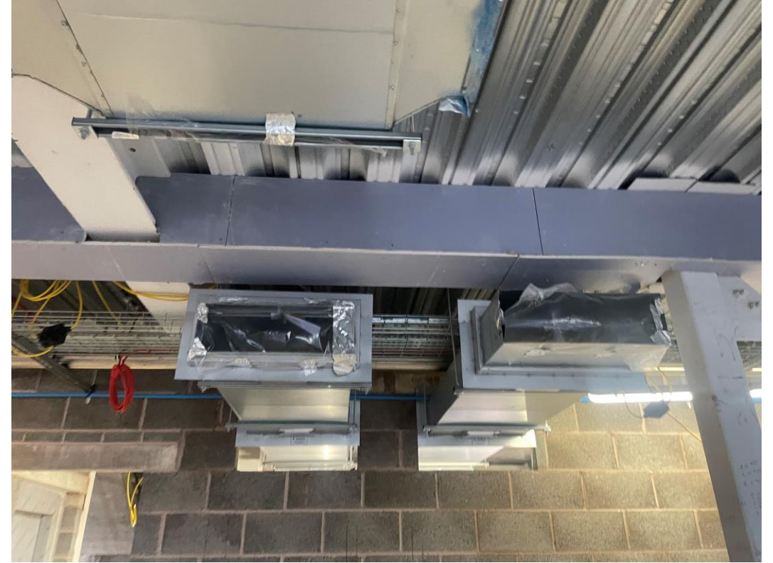
Residential Block – Mechanical ducting installation on-going
