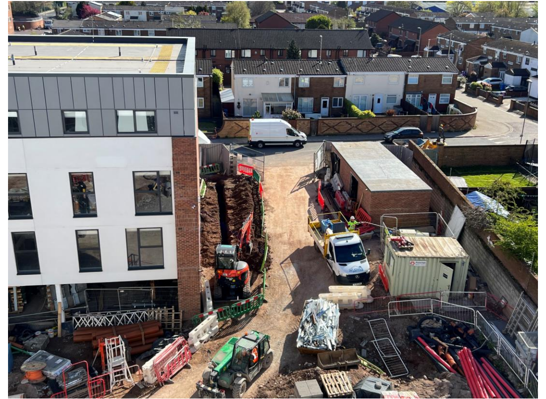
Excavation commenced for water connection
