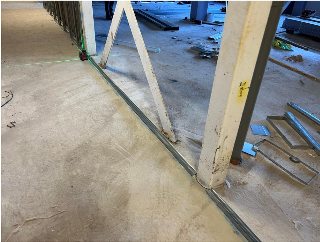
Residential Block – Setting out of partitions on-going
