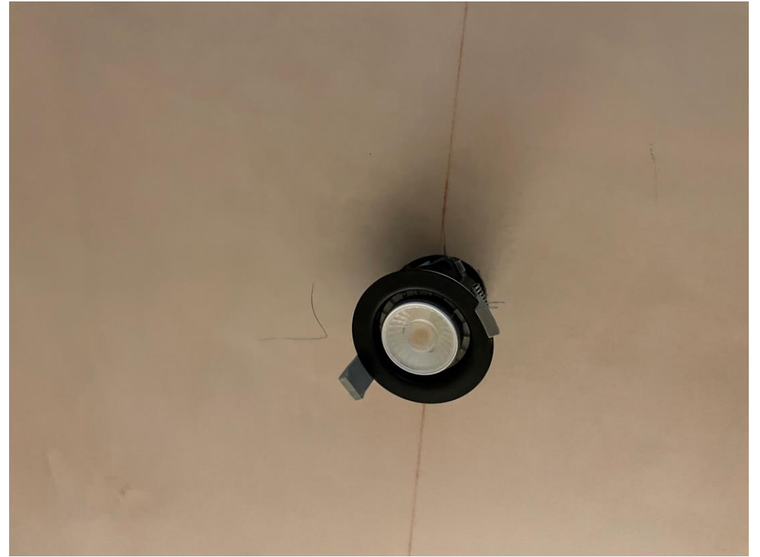
Residential Block – Light fitting installation commenced
