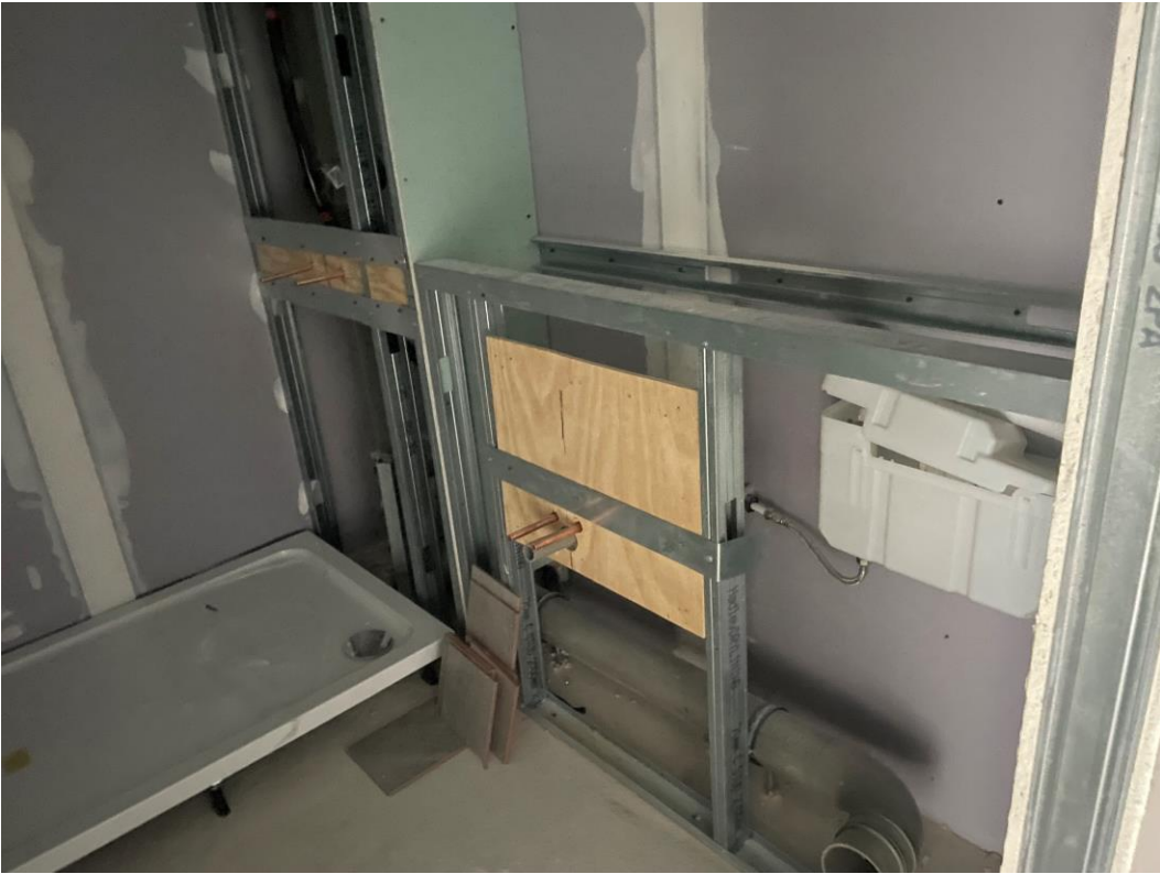
Residential Block – IPS Installed
