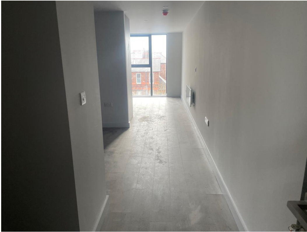
Residential Block – Apartment finishes
