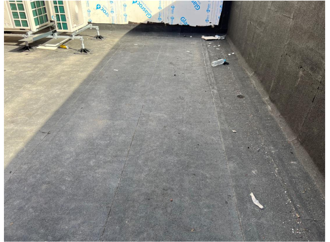
Residential Wing – Felt parapet upstand
