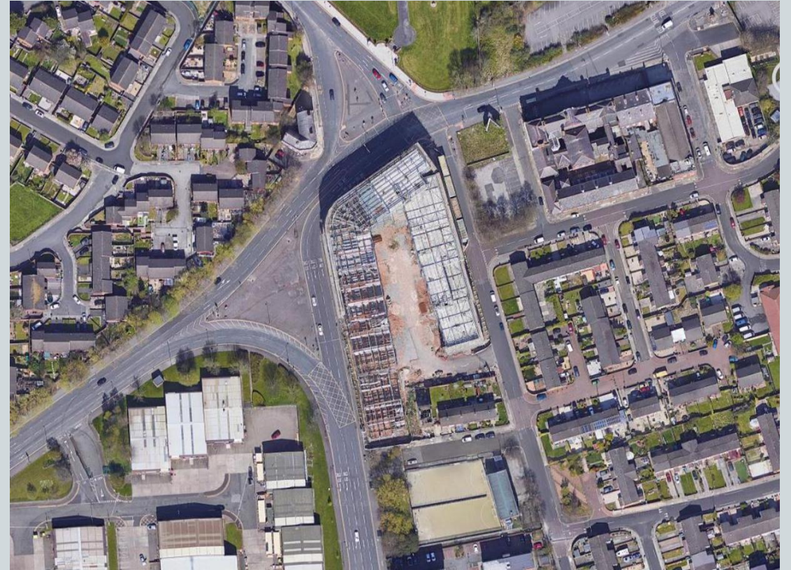
Aerial view of Element – The Quarter site location
