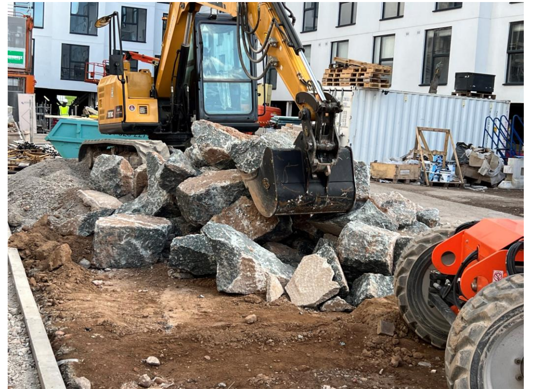
Excavations for water connection on-going
