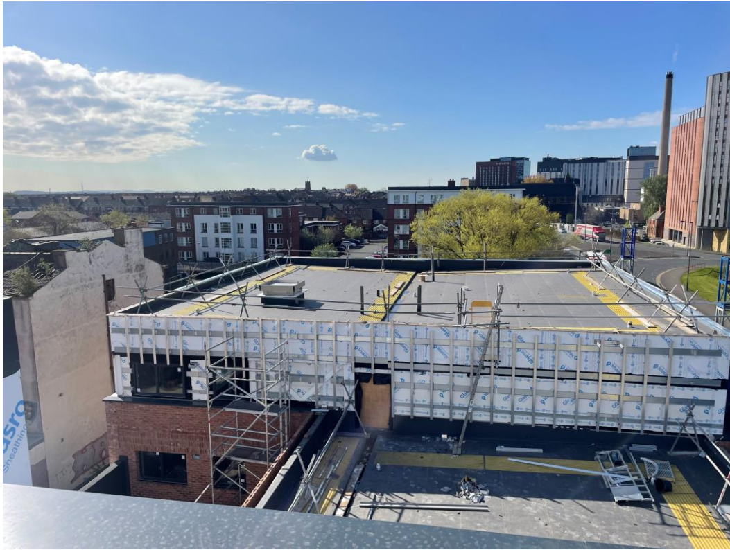
Commercial Block – Weatherboarding installation complete
