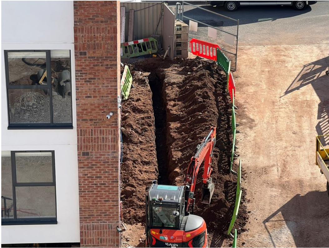
Excavation commenced for water connection
