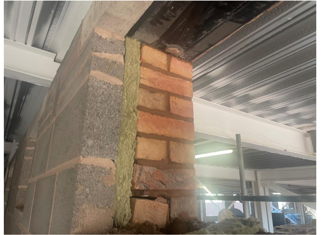
Residential Wing - Brick & block cavity wall construction
