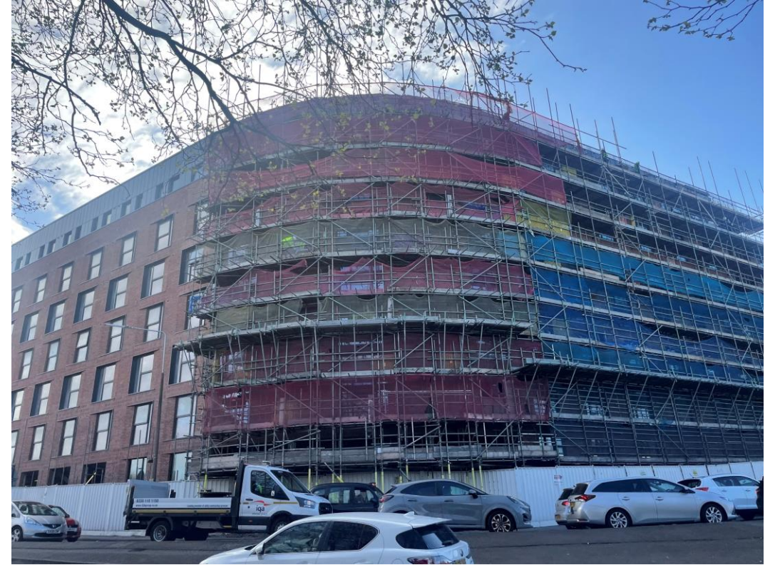
West Derby Road - Site view
