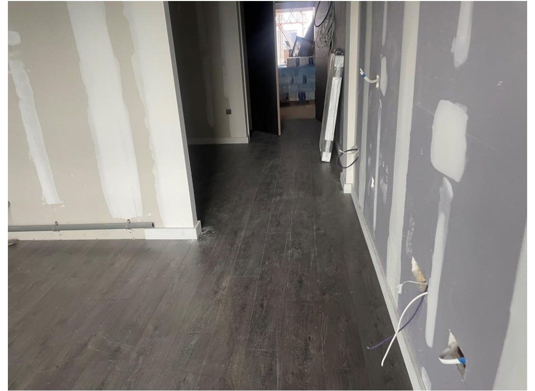
Residential Block – Laminate flooring installed
