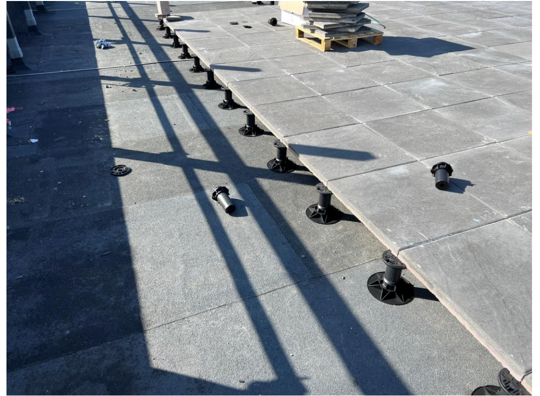
Residential Wing – Paving installation commenced
