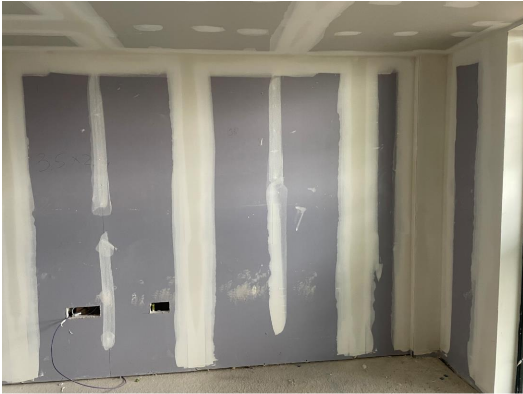
Residential Block – Internal walls boarded, taped and jointed
