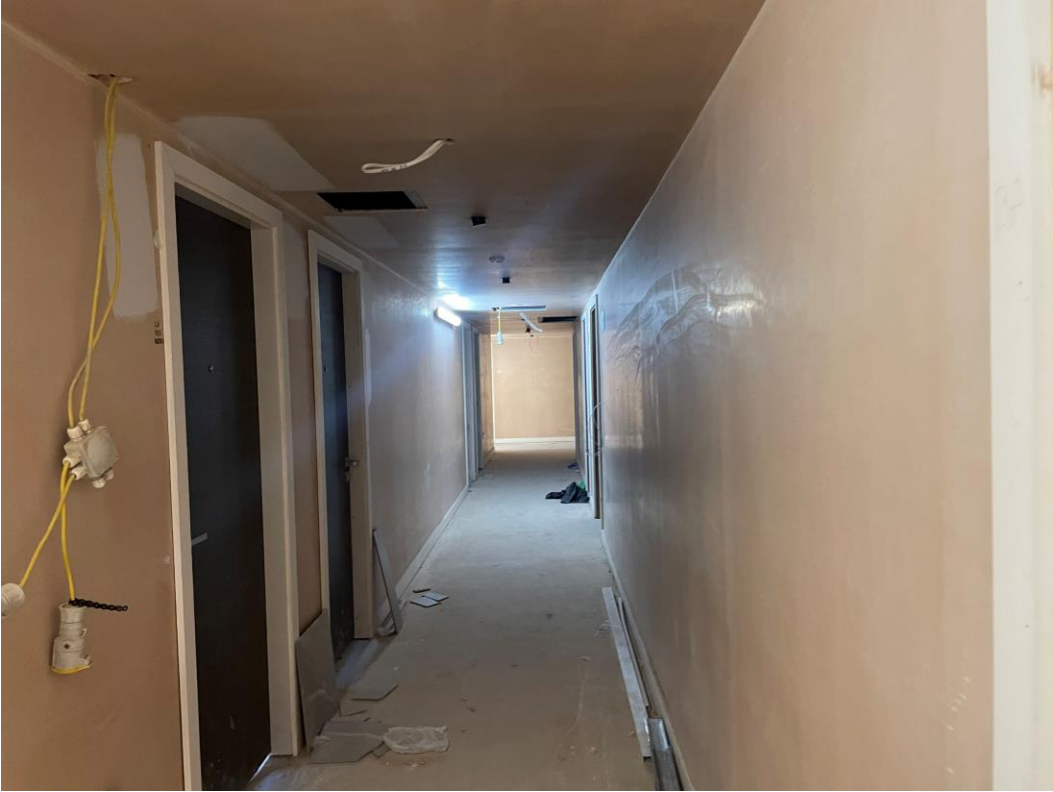
Residential Block – Walls & ceilings plastered
