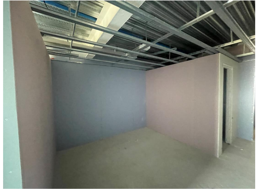
Residential Block – Metal partition erection and boarding
