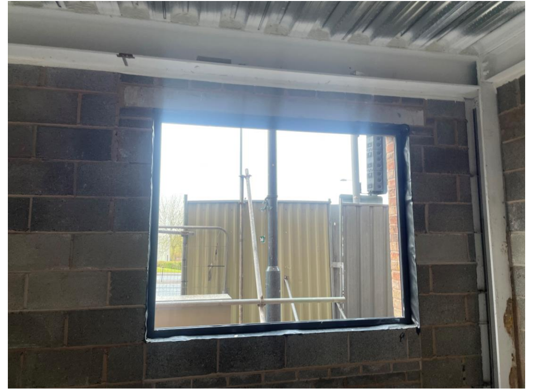
Residential Block – Window unit installation on-going
