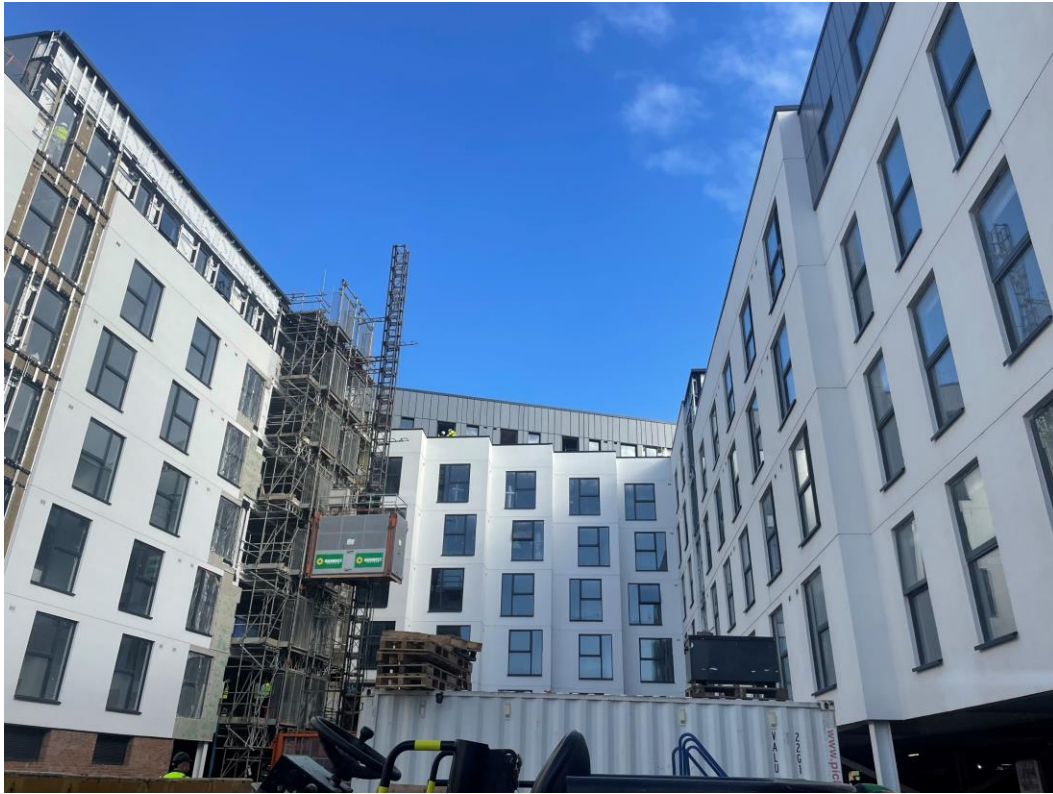
Residential Block – Viewed from site court yard
