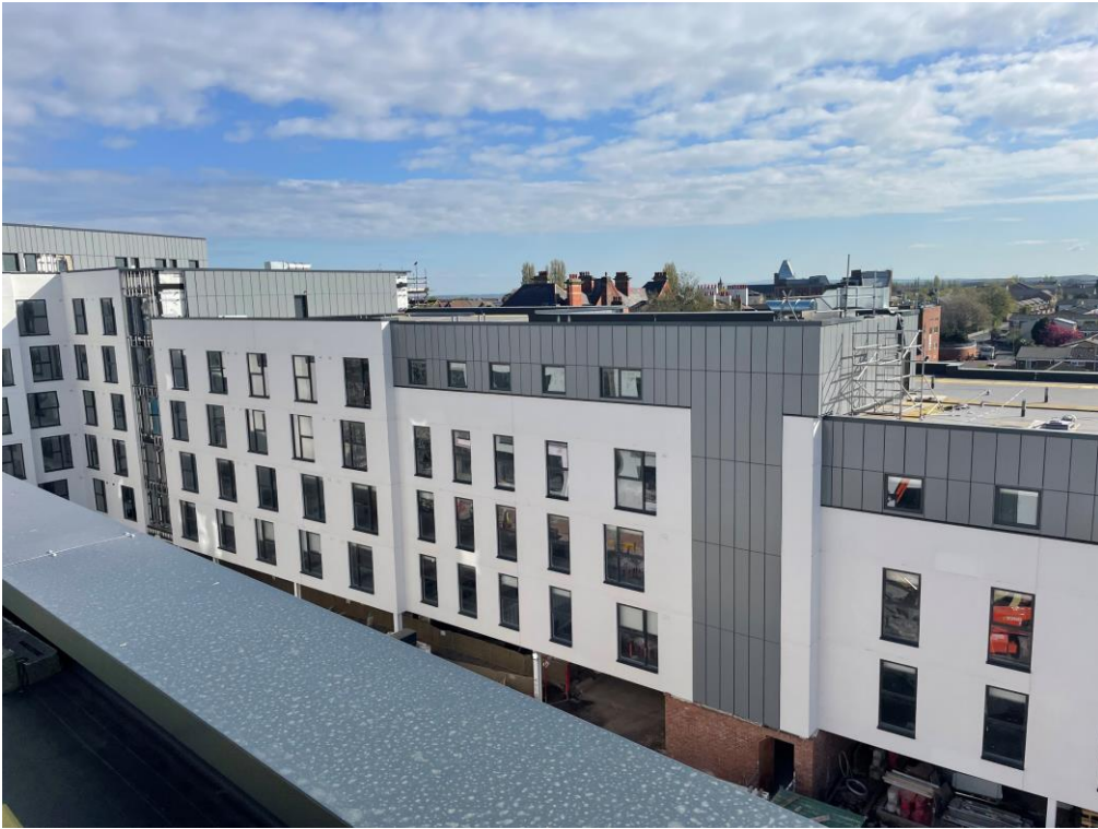
Cladding installation on-going
