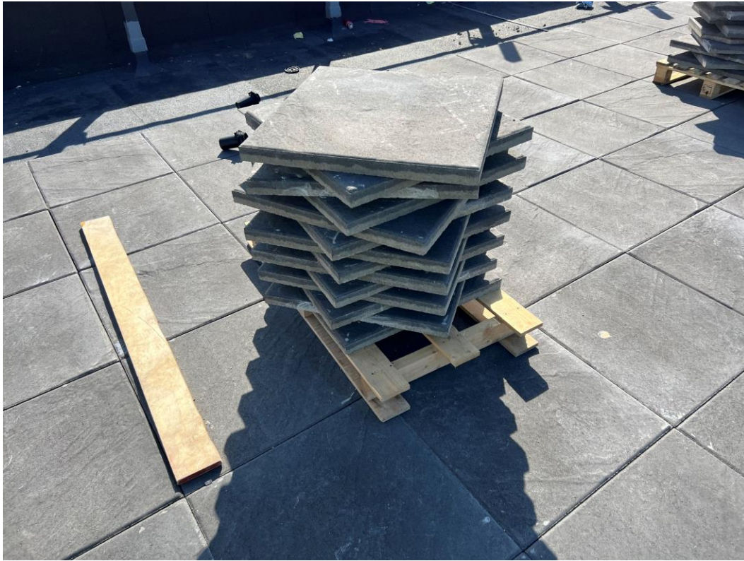
Residential Wing – Paving installation commenced
