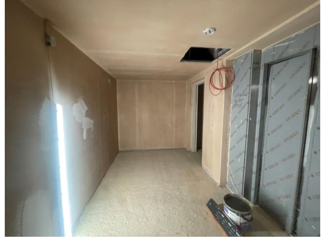
Student Block – Lift lobby walls & ceiling plastered
