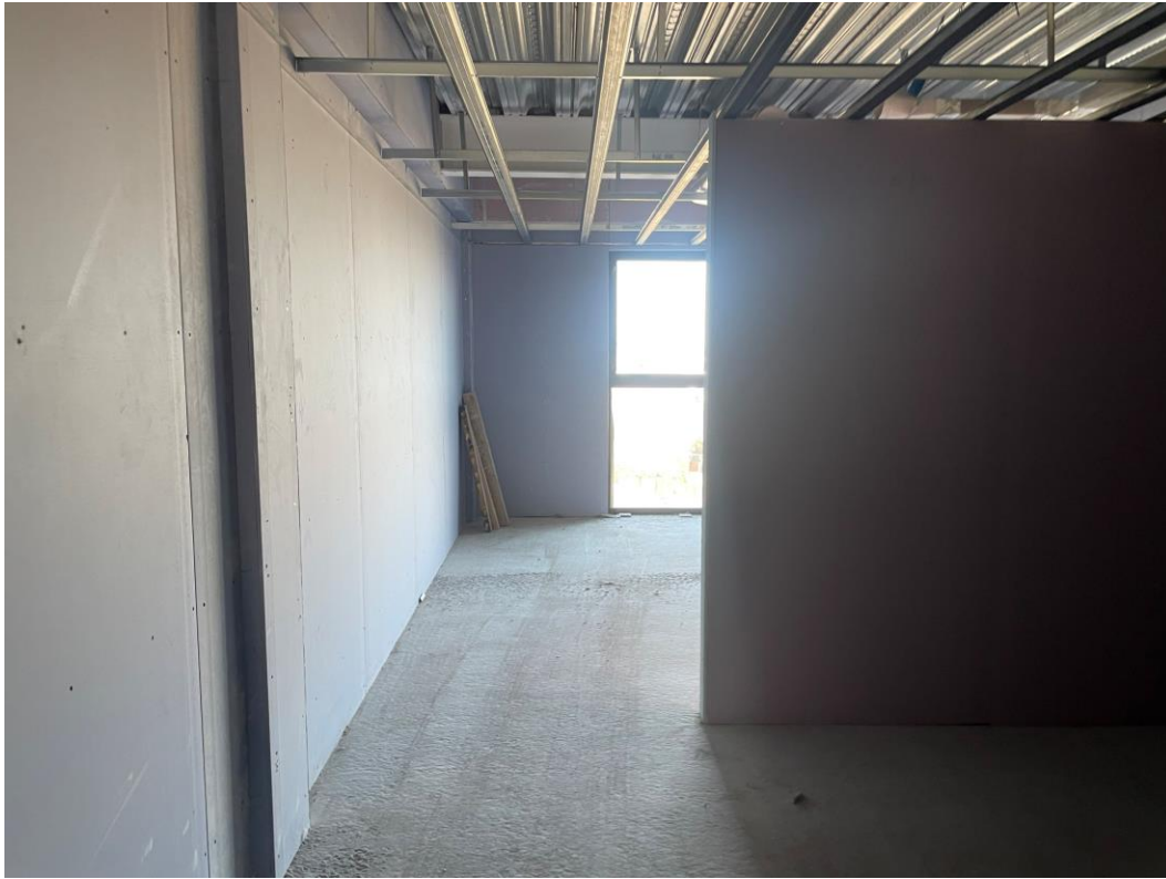
Residential Wing – Partitions erected and boarded
