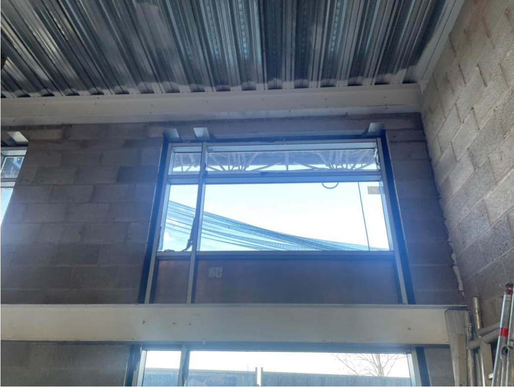
Commercial Block – Curtain walling installation on-going
