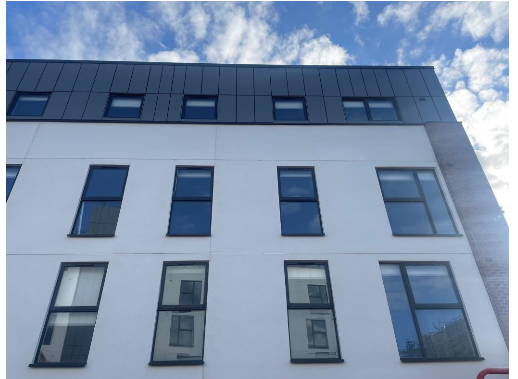
Cladding installation on-going
