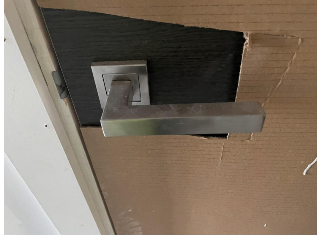
Student Wing – Ironmongery installation
