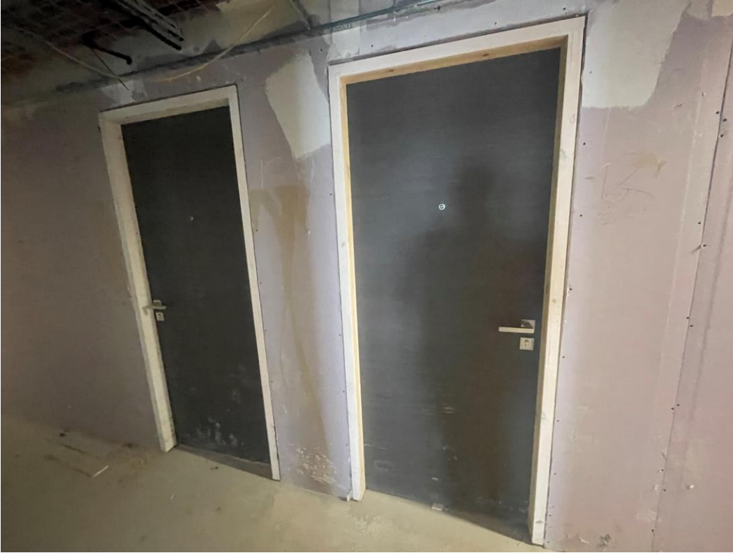
Student Wing – Apartment doors installed
