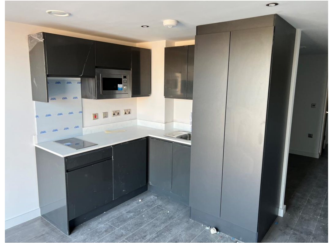
Residential Block – Kitchen complete
