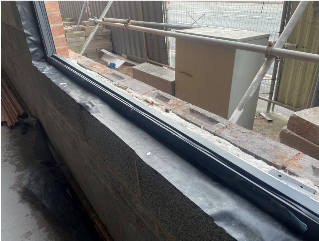
Residential Block – Window unit installation on-going
