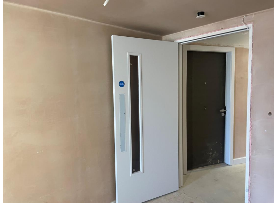
Student Wing – Installation of doors on-going
