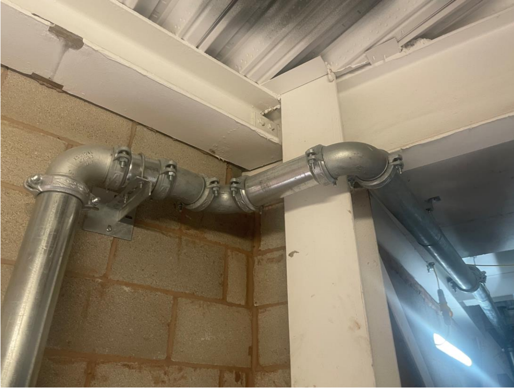
Residential Block – Dry Riser installation on-going
