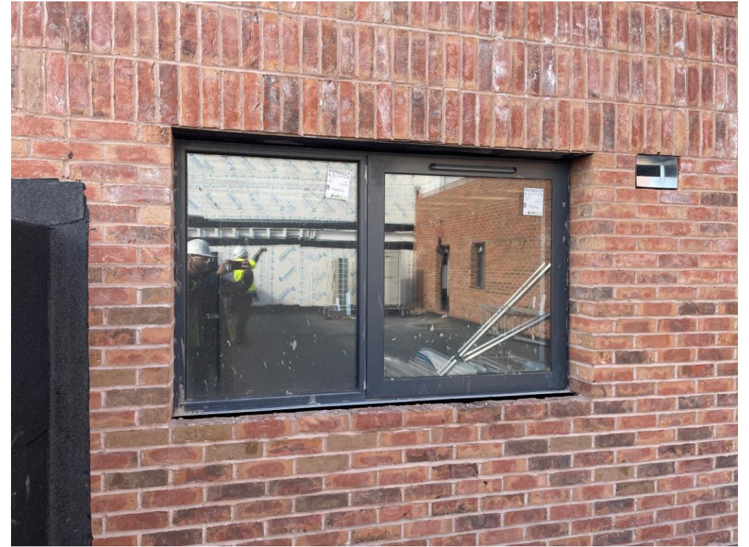
Window installation on-going
