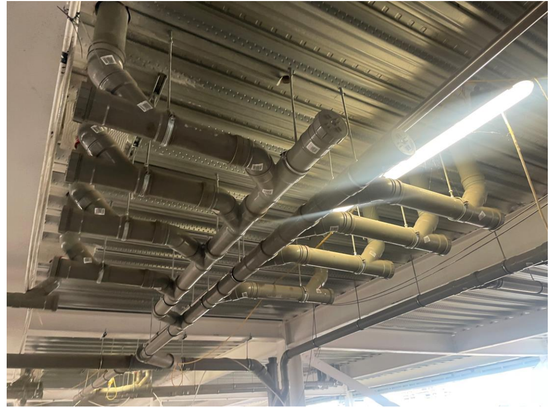
Residential Wing – Apartment drainage
