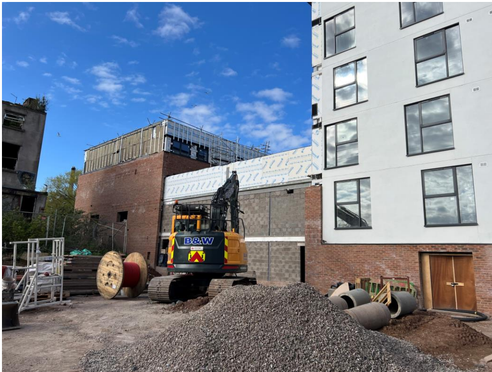
Commercial Units – Scaffolding removal complete
