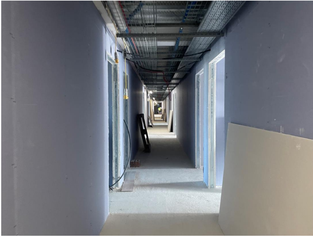
Residential Block – Metal partitions insulation and boarded
