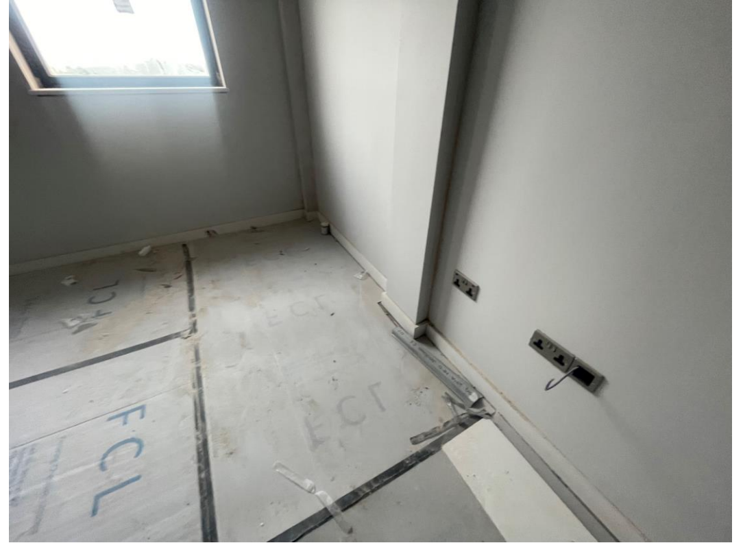
Residential Block – Laminate & skirting board installation
