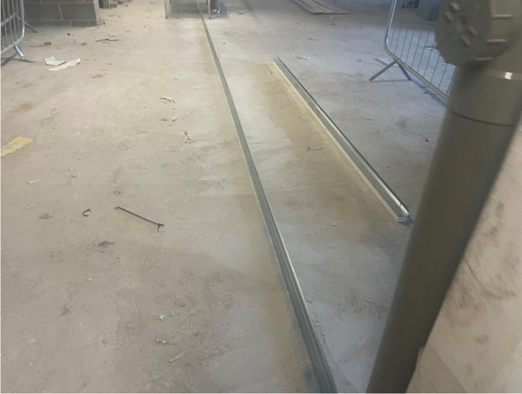
Ground Floor – Setting out of partitions
