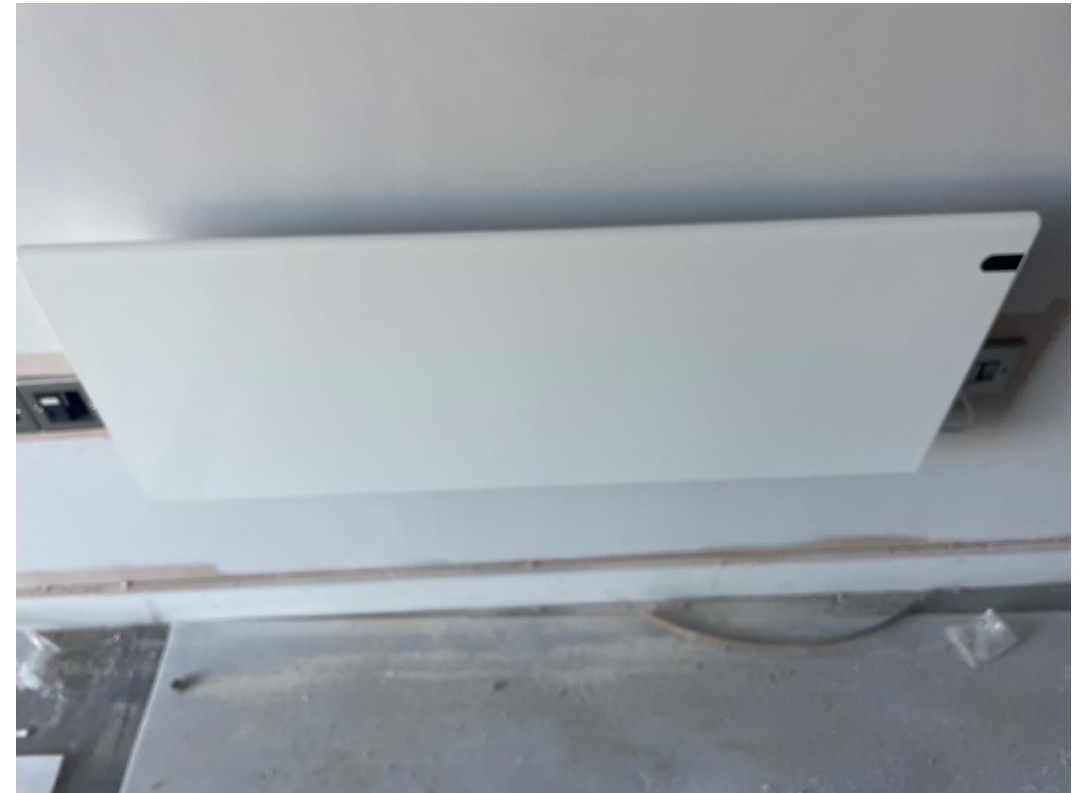
Residential Block – Radiator installation
