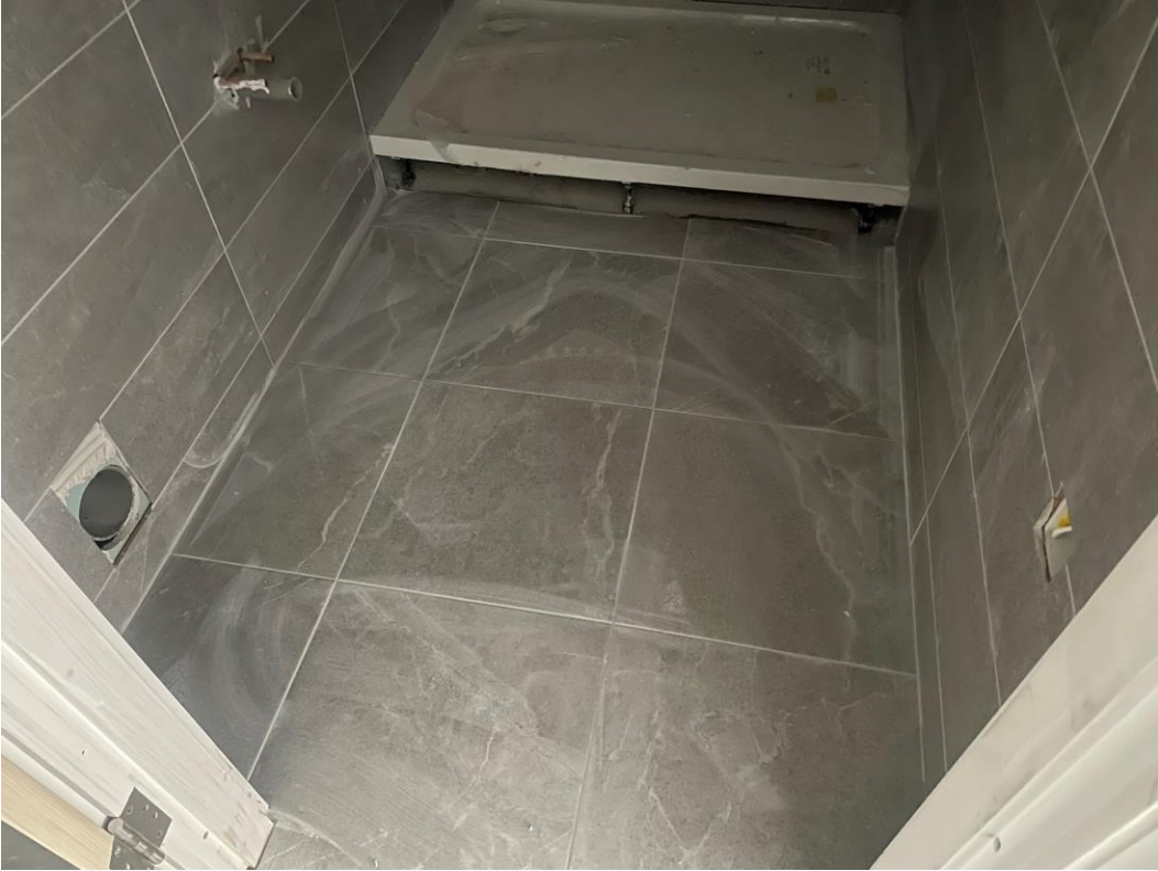
Residential Block – Floor tiles installed
