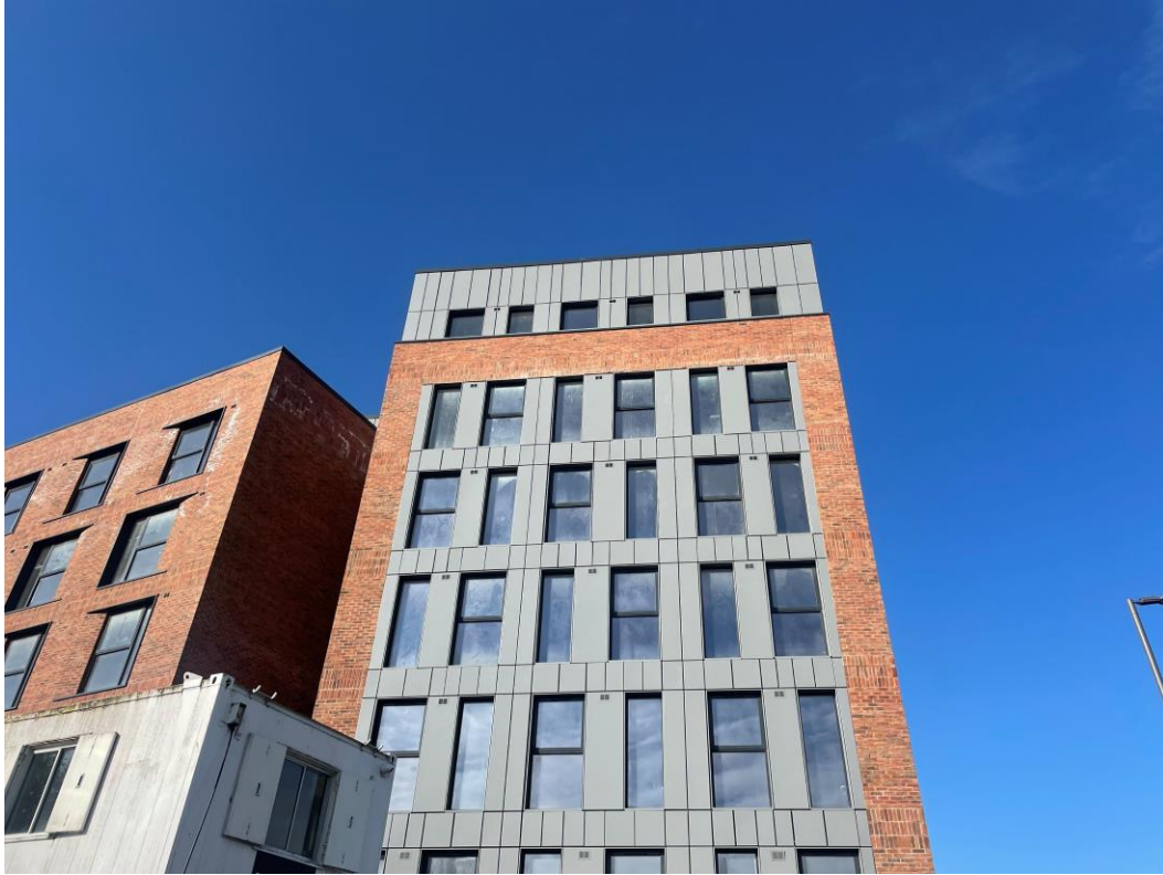
West Derby Road - Site view
