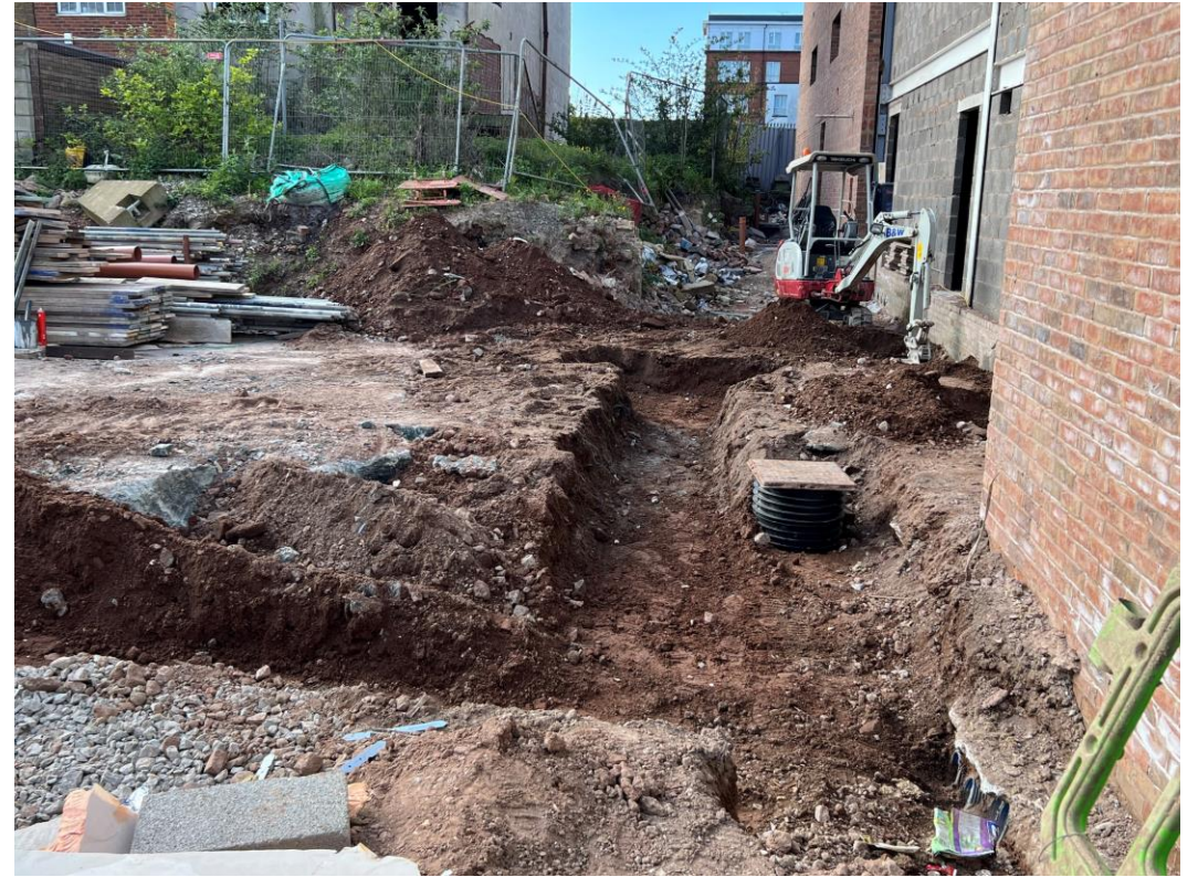
Excavations on-going for services connection
