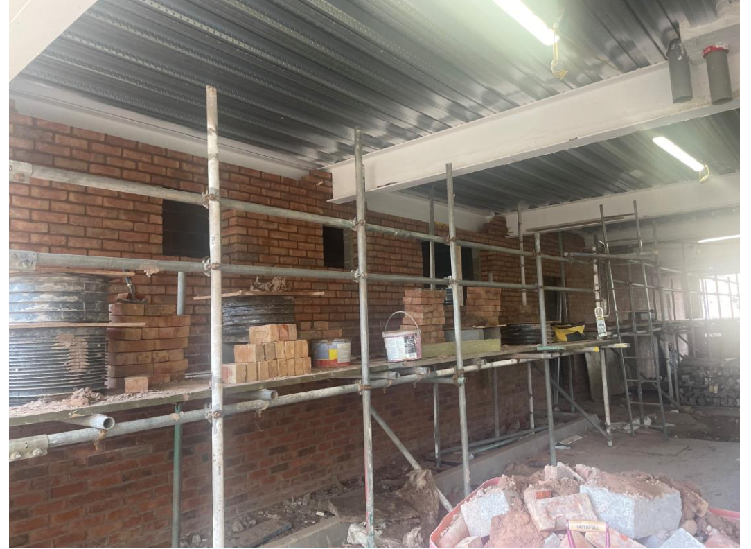
Commercial Block – Internal brickwork on-going
