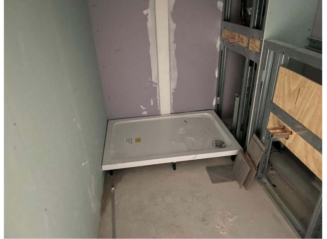
Residential Block – Shower tray installed
