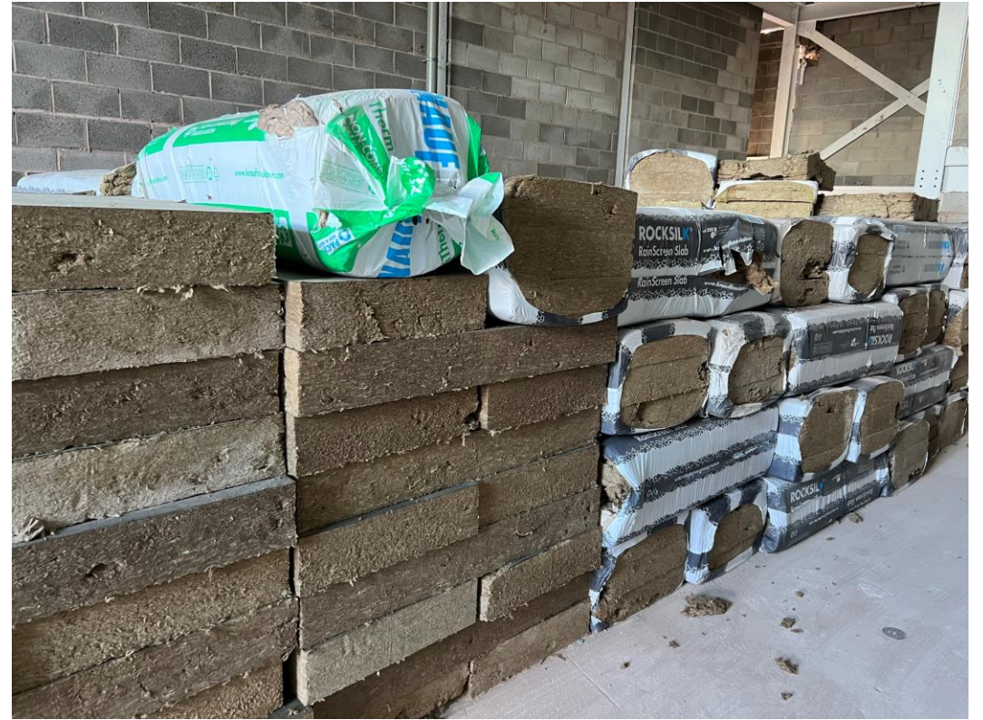
Material Storage – Knauf soffit Insulation
