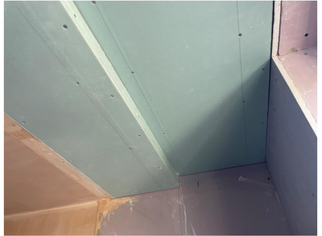
Student Wing – Ceilings boarded and skimmed
