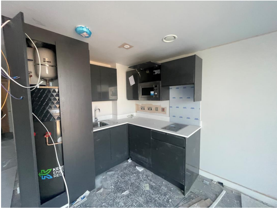
Student Wing – Kitchen installation
