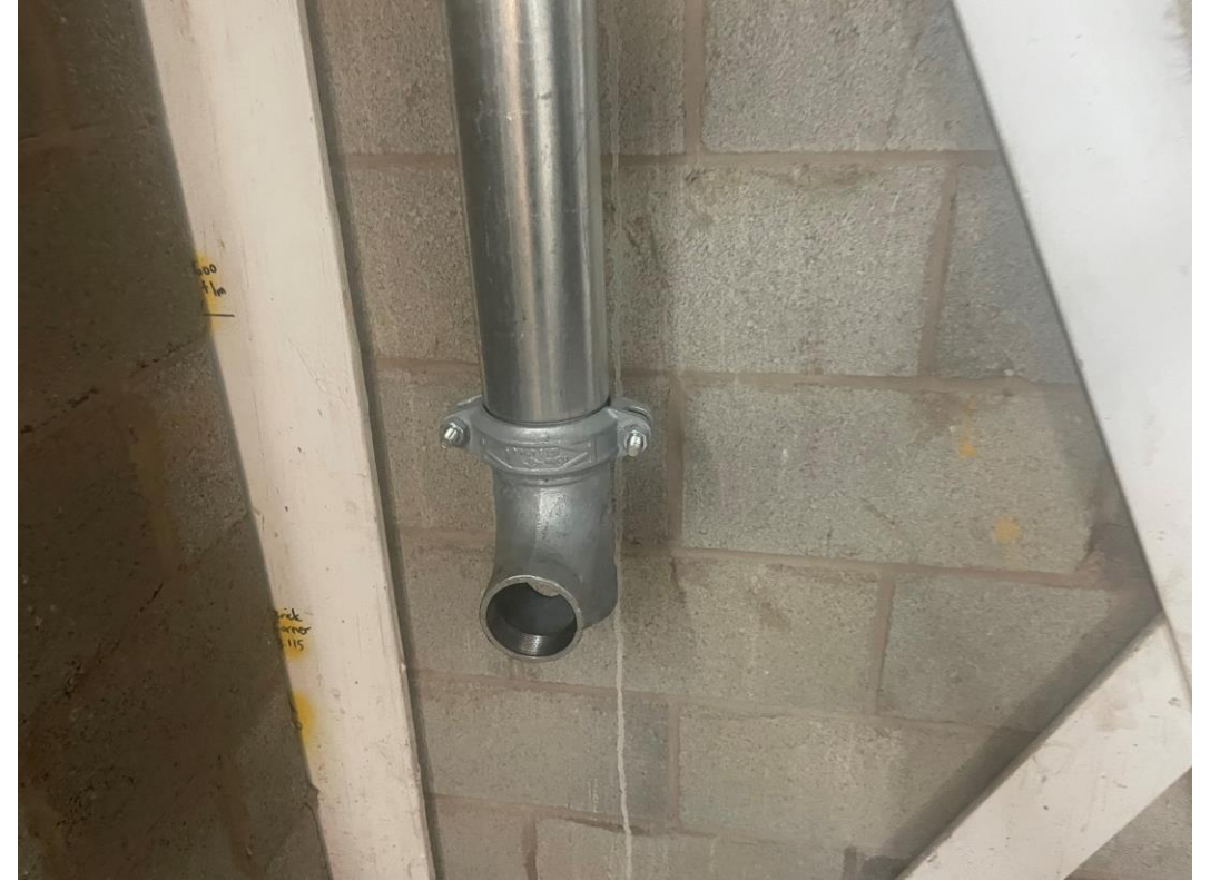
Residential Block – Dry Riser installation on-going
