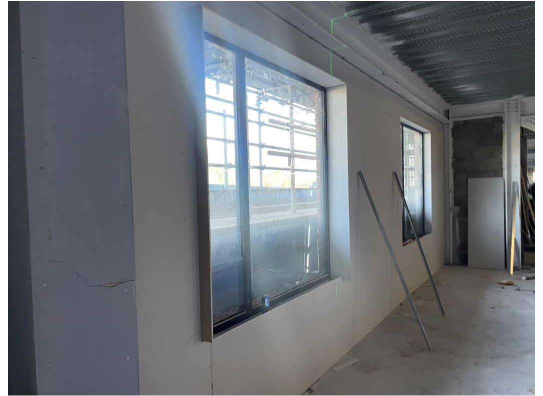
Residential Block – Boarding out of window wall
