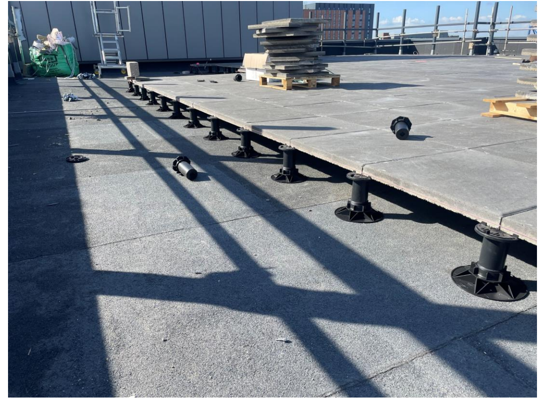
Residential Wing – Paving installation commenced
