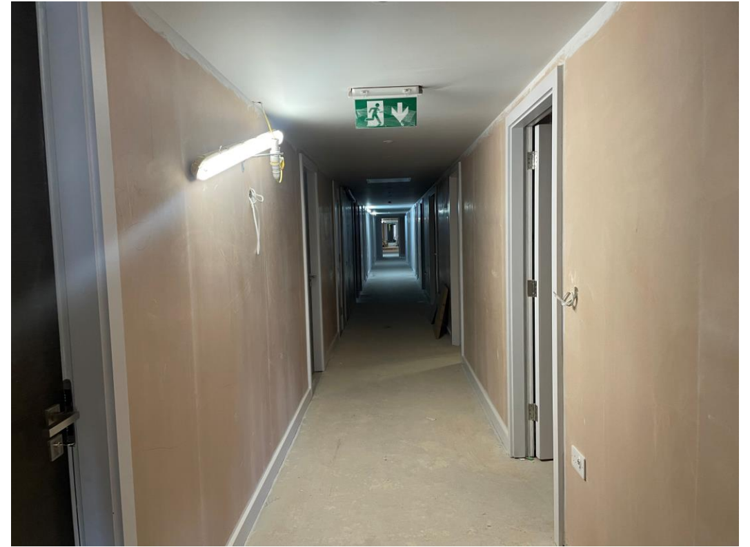
Student Wing – Walls & ceilings plastered
