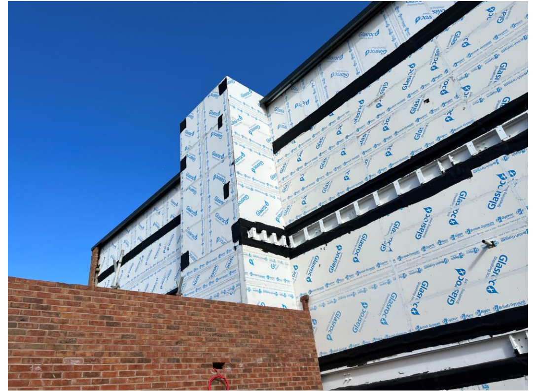
Residential Block – Weatherboarding installation complete
