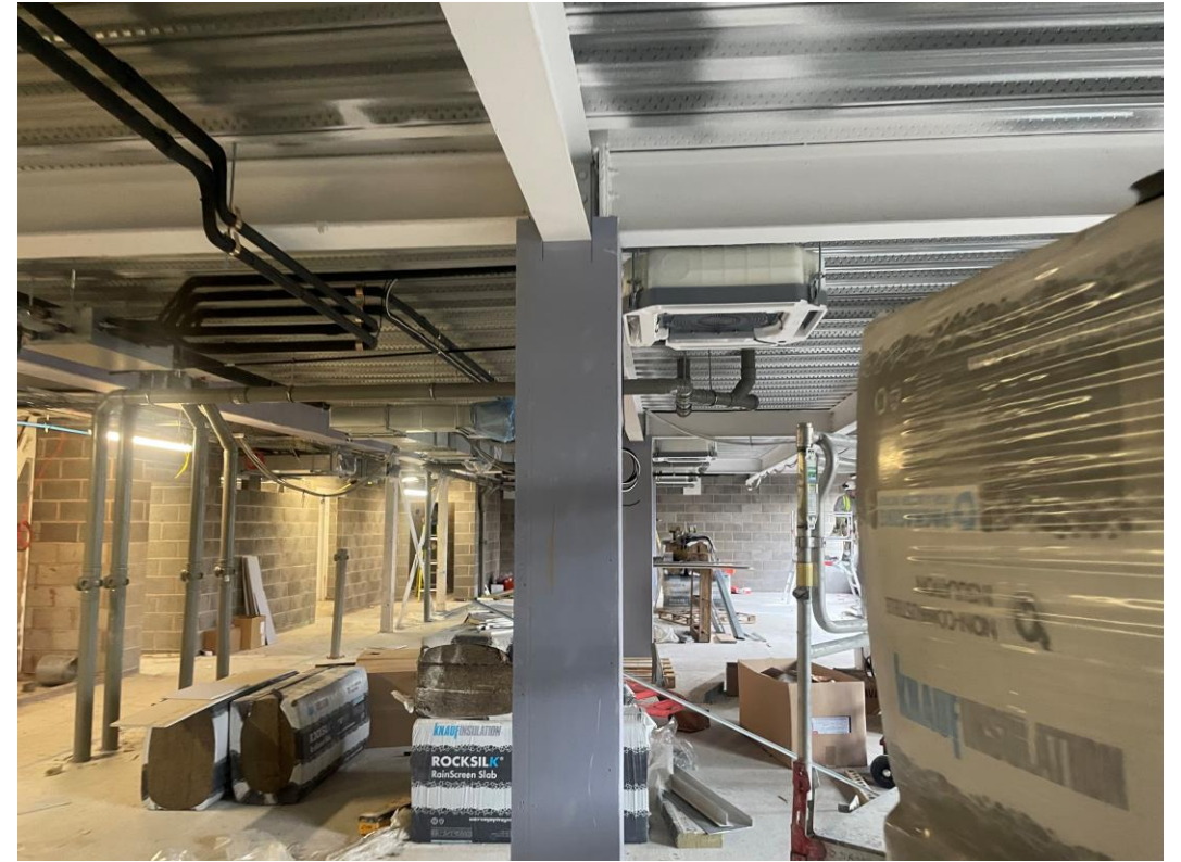
Residential Block – Boarding of steel components
