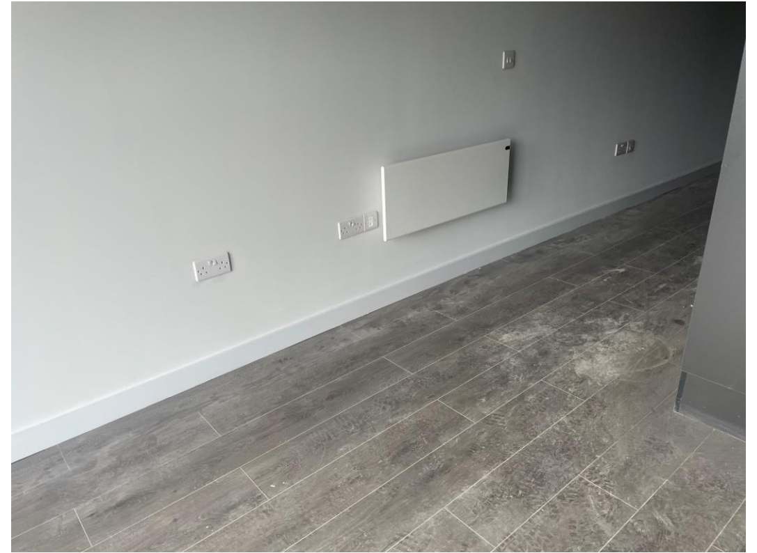
Residential Block – Apartment finishes
