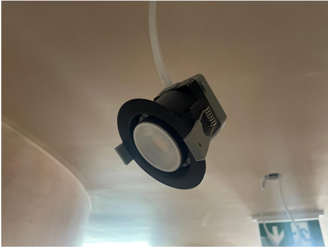
Residential Block – Light fitting installation commenced
