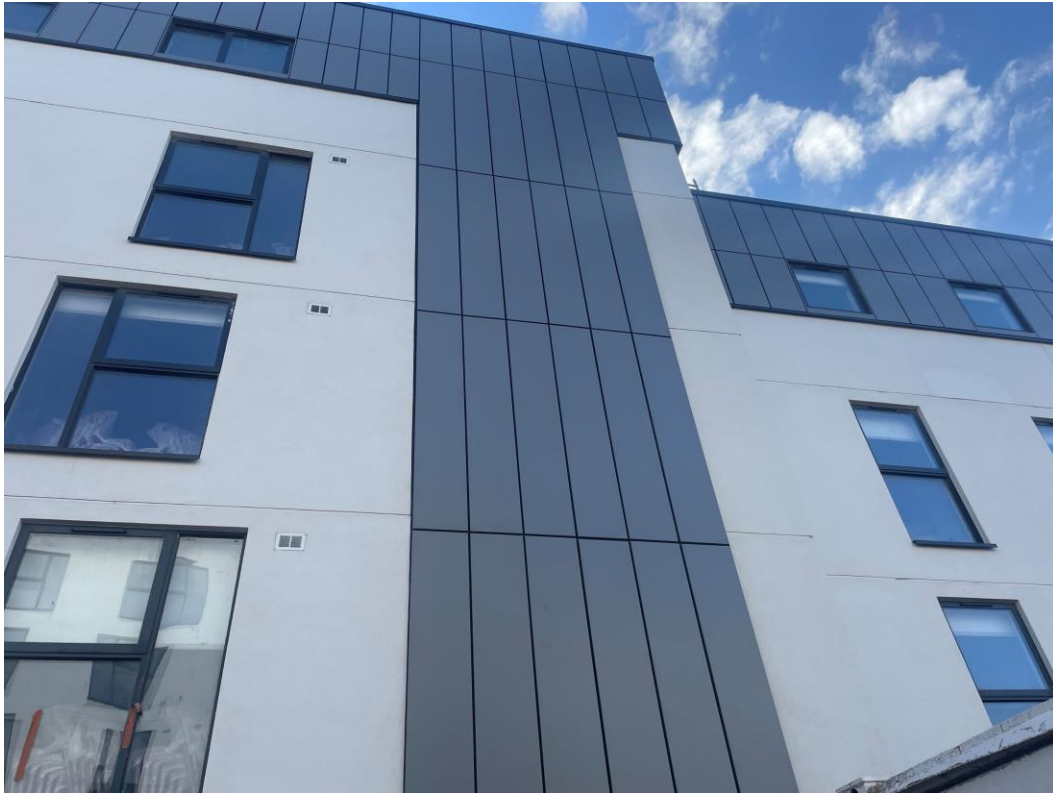
Student Wing – Cladding installation on-going
