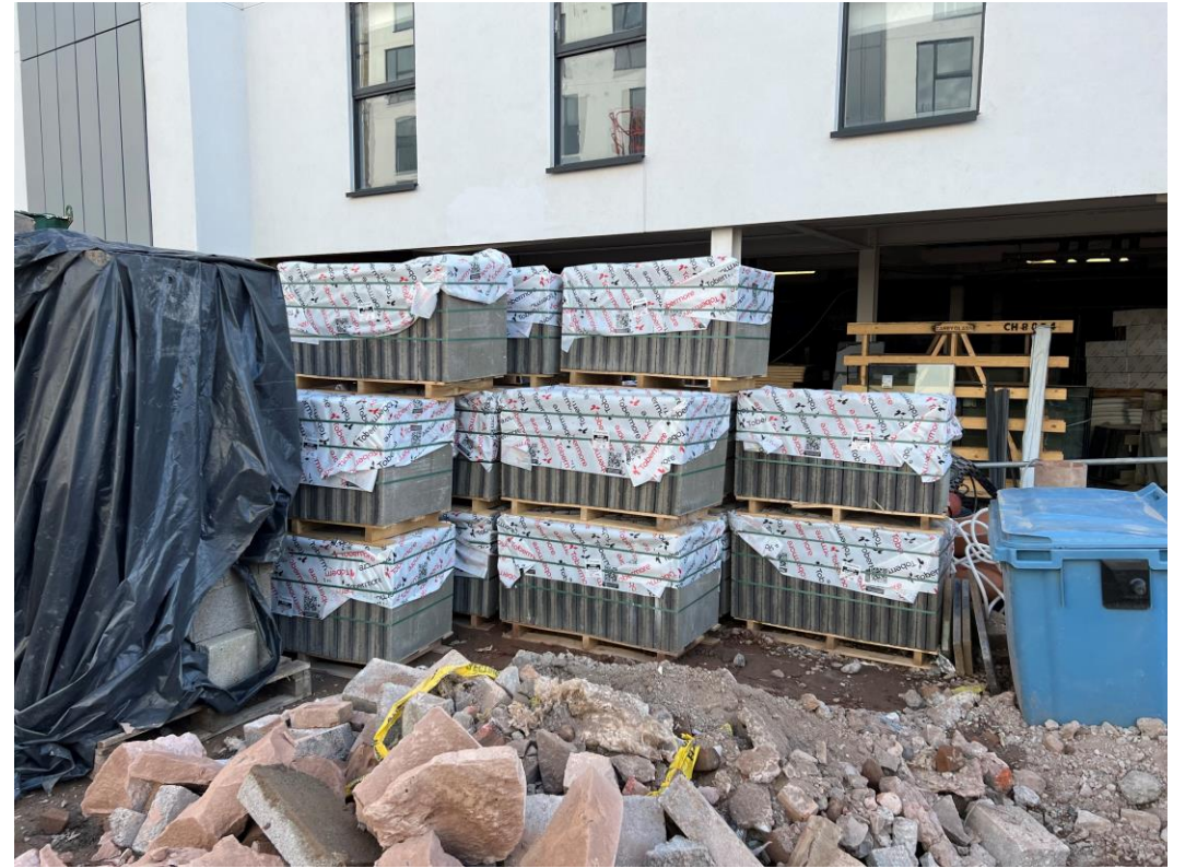
Materials Stored – Paving slabs
