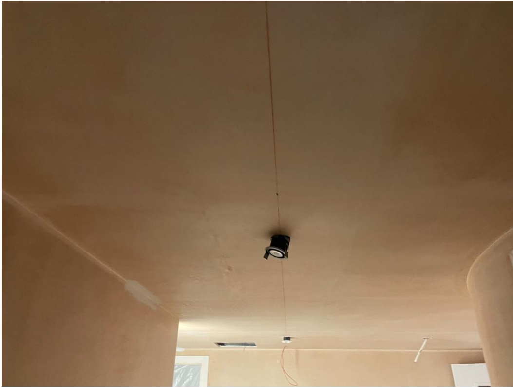
Residential Block – Light fitting installation commenced
