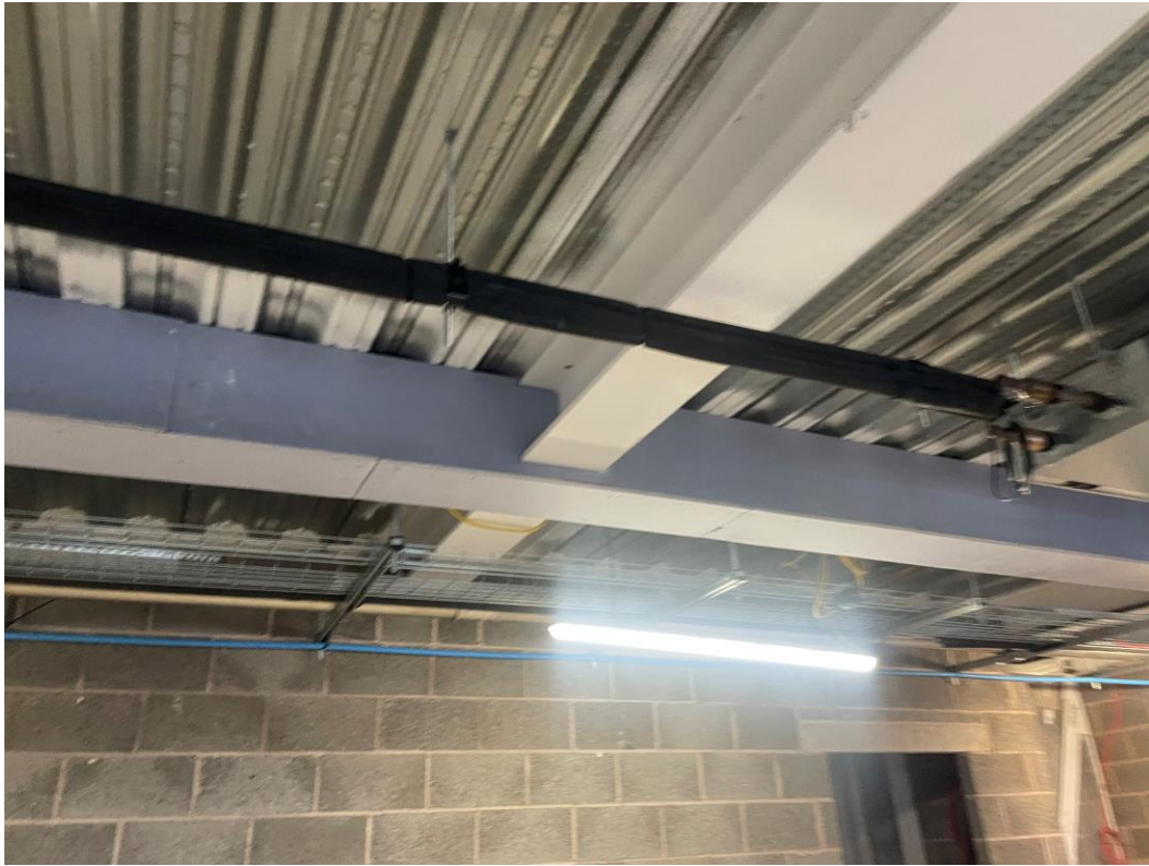
Residential Block – Boarding of steel components
