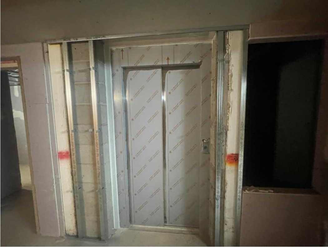
Student Block – Metal framework installation commenced to lift
