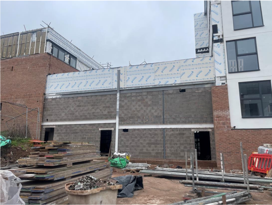
Commercial Block – Scaffolding removal nearing completion
