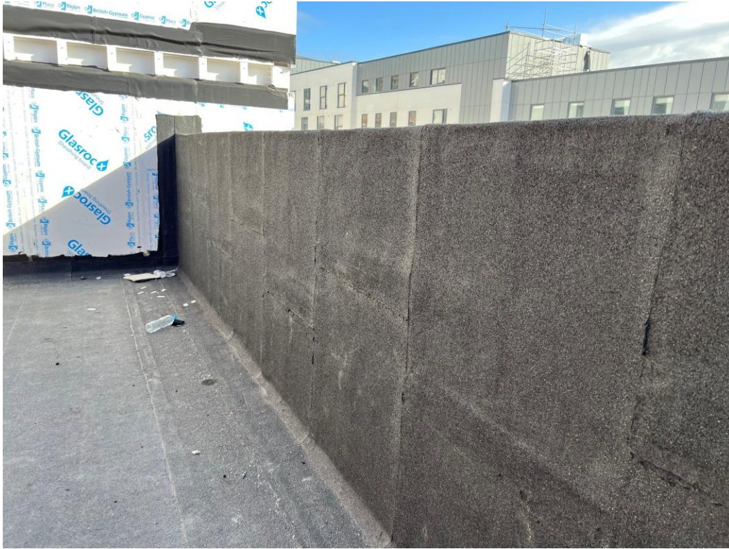
Residential Wing – Felt parapet upstand
