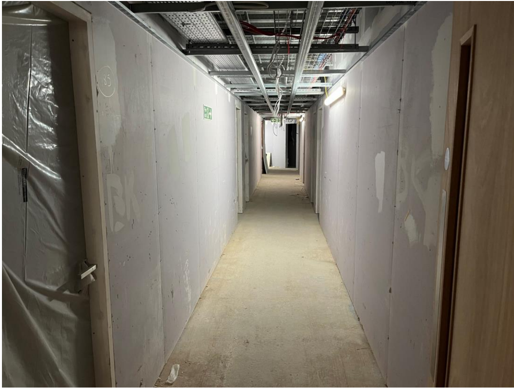
Student Wing – Internal finishes on-going
