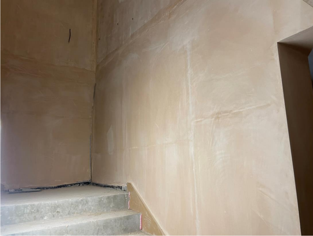
Residential Block – Plastering to stair cores on-going
