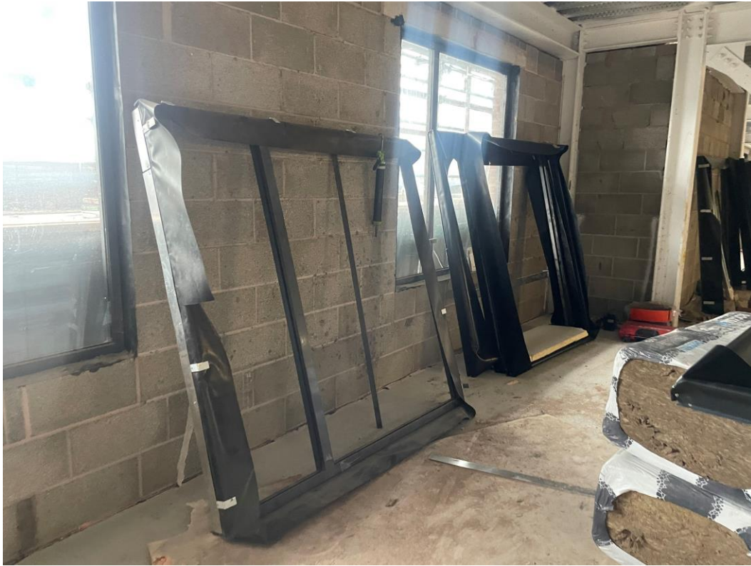
Material Storage – Window units
