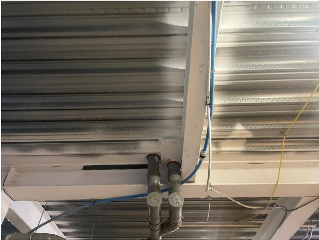
Student Wing – Internal drainage and fire stopping on-going
