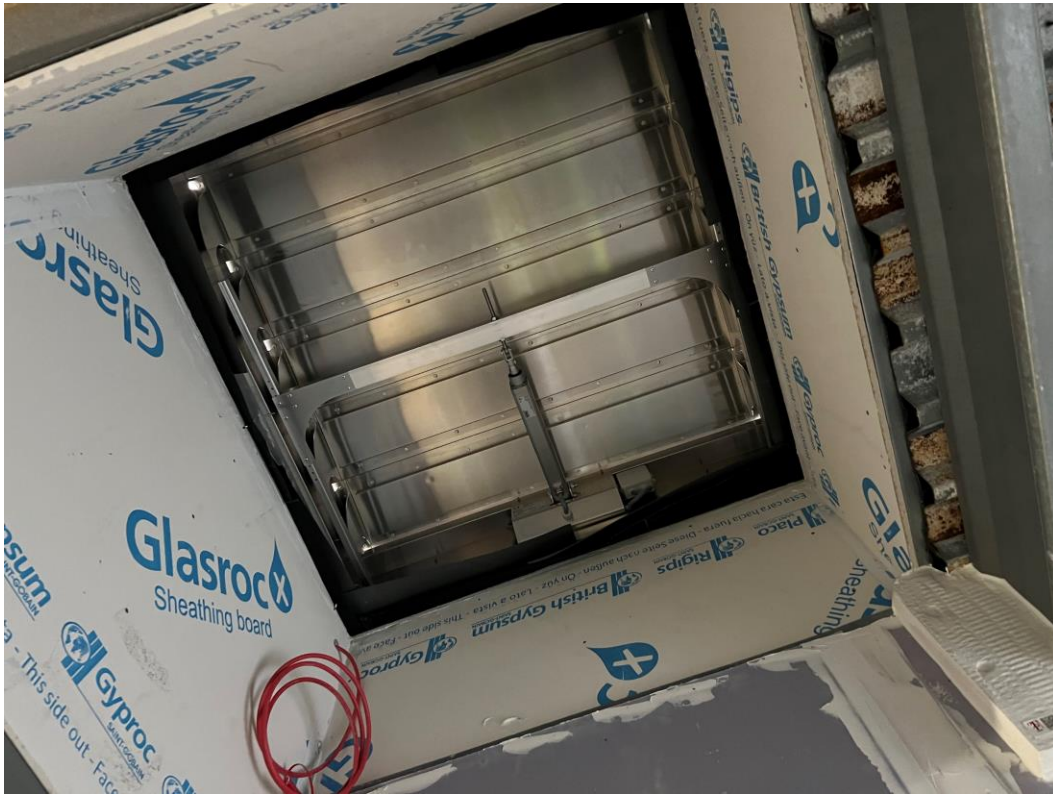
Residential Wing – AOV Installation on-going
