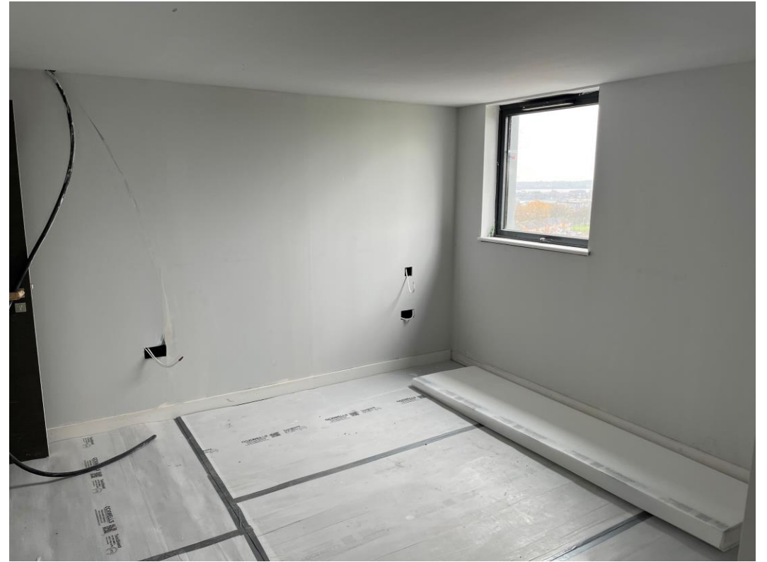
Student Block - Internal finishes on-going
