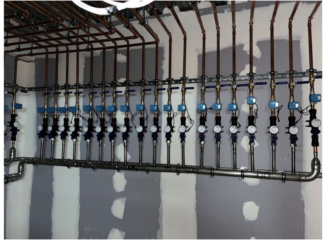
Student Wing – Water meters installed
