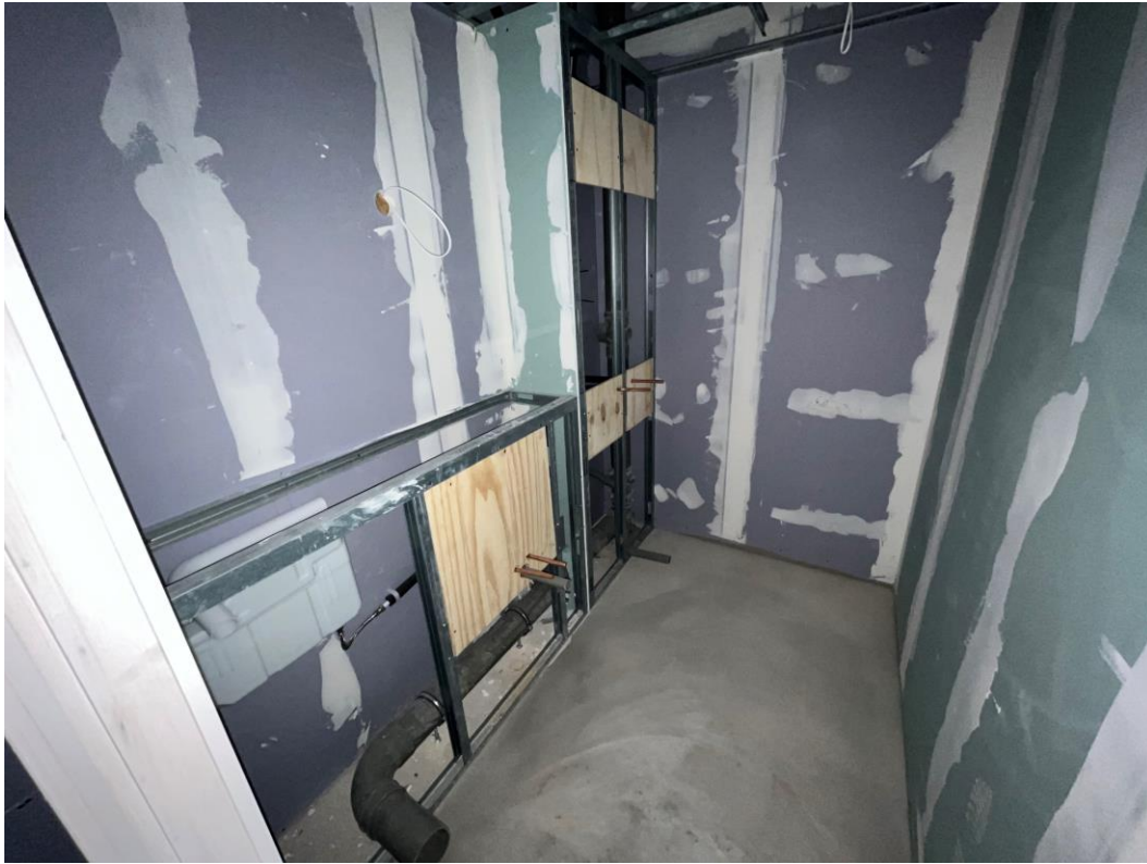
Residential Block – IPS Installed
