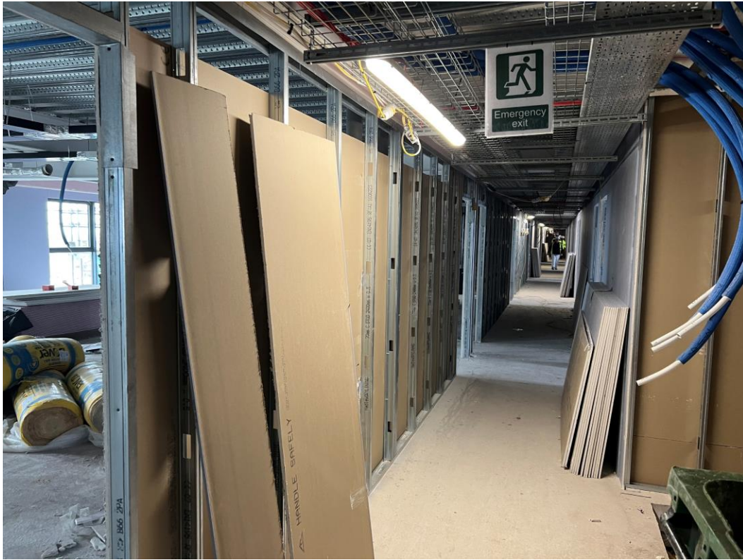
Residential Block – Metal partition erection
