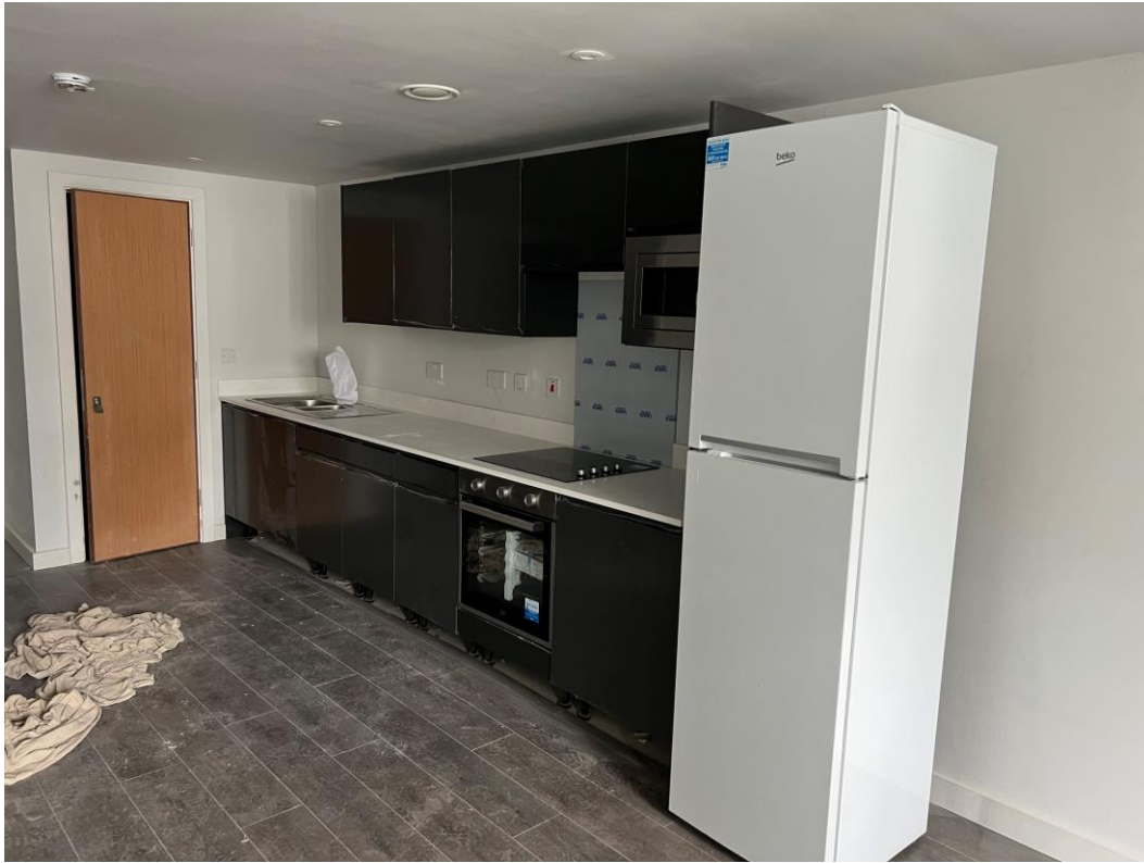
Student Wing – Kitchen installation
