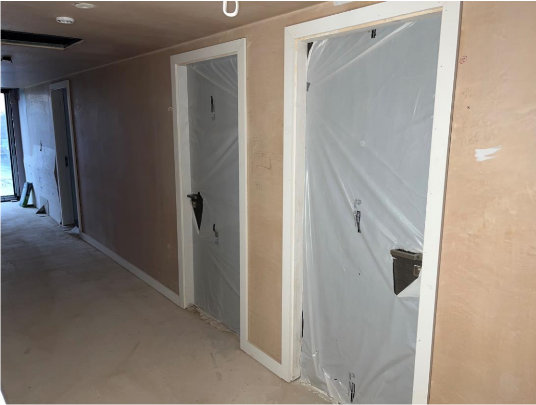
Student Wing – Apartment doors installed
