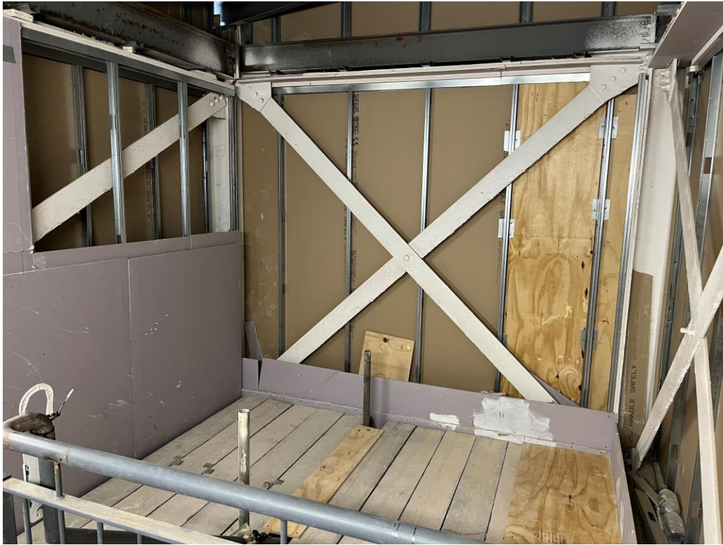
Residential Block – Pattress installation and boarding of stair core walls
