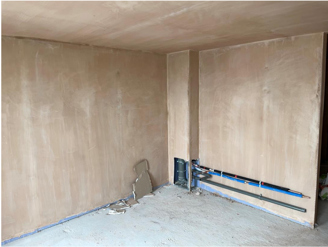
Student Block – Plastering on-going
