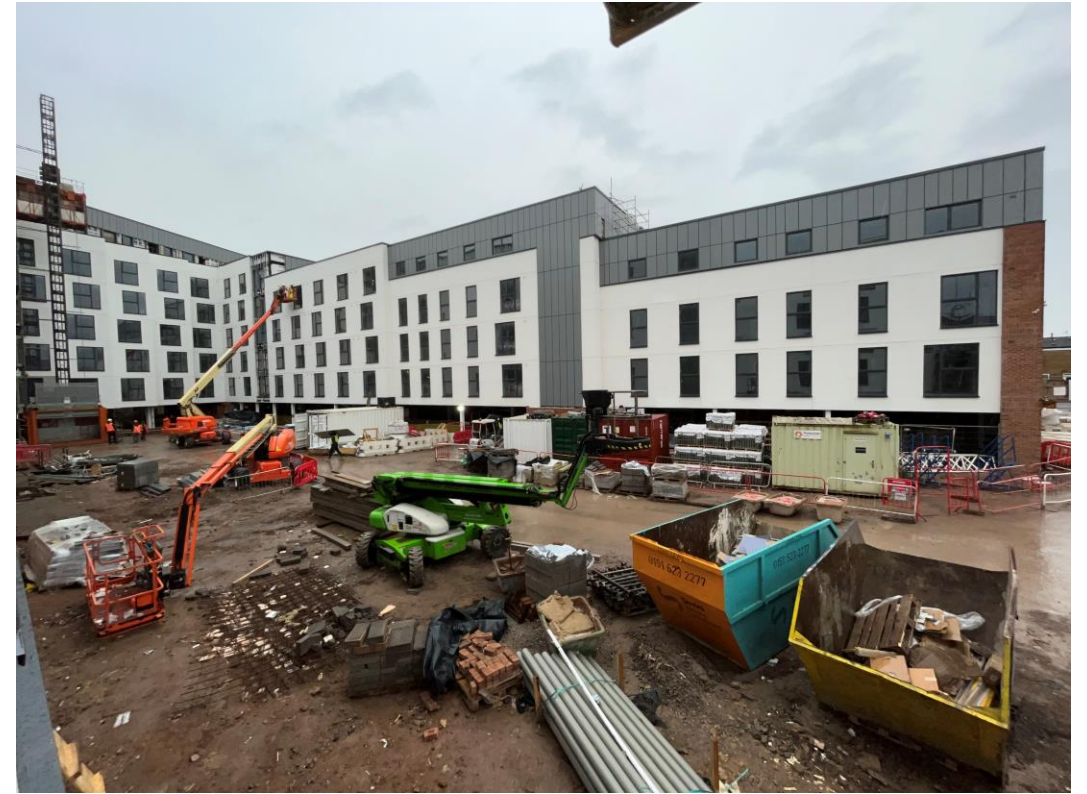
Student Wing – Cladding installation on-going
