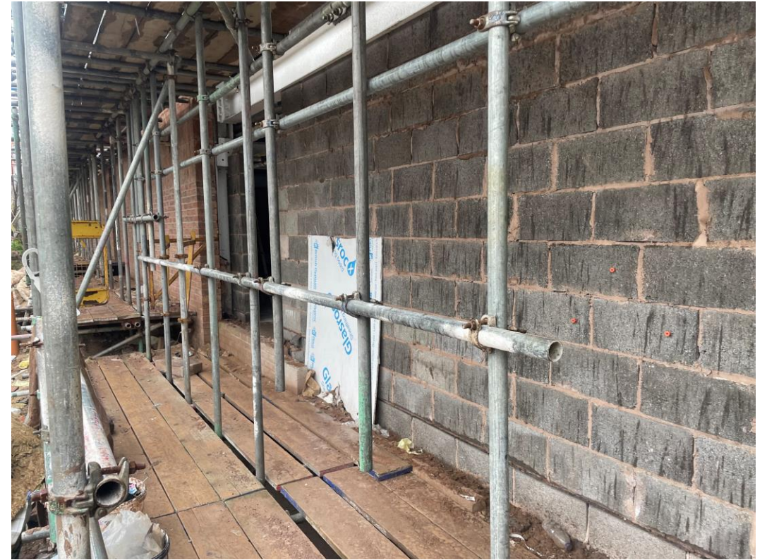
Commercial Block – Scaffolding and External blockwork on-going
