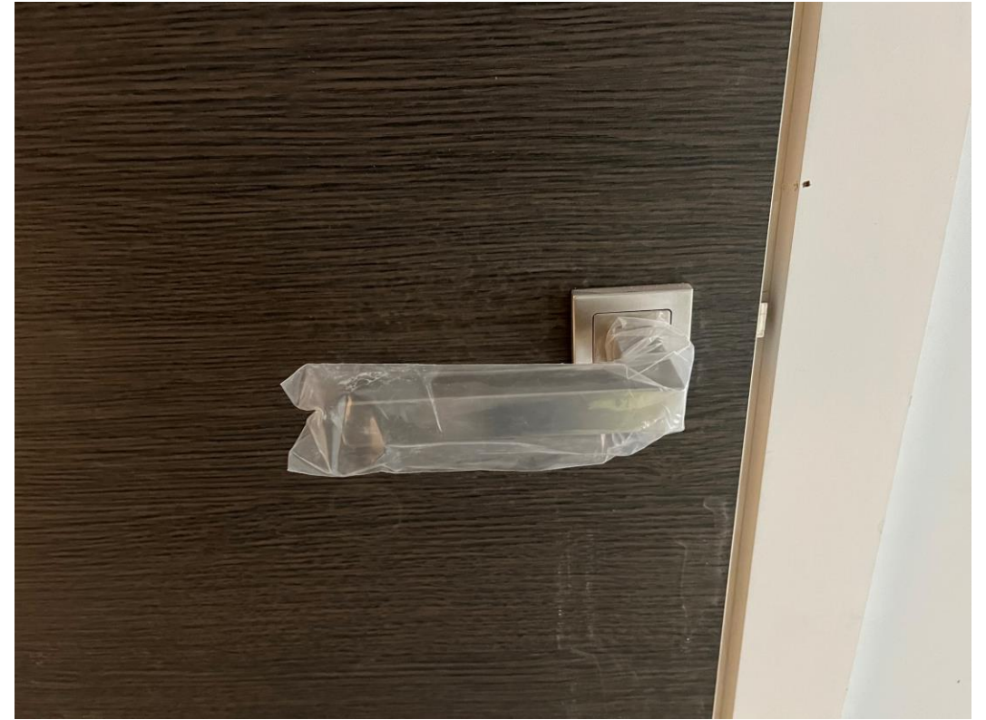
Student Wing – Ironmongery installation
