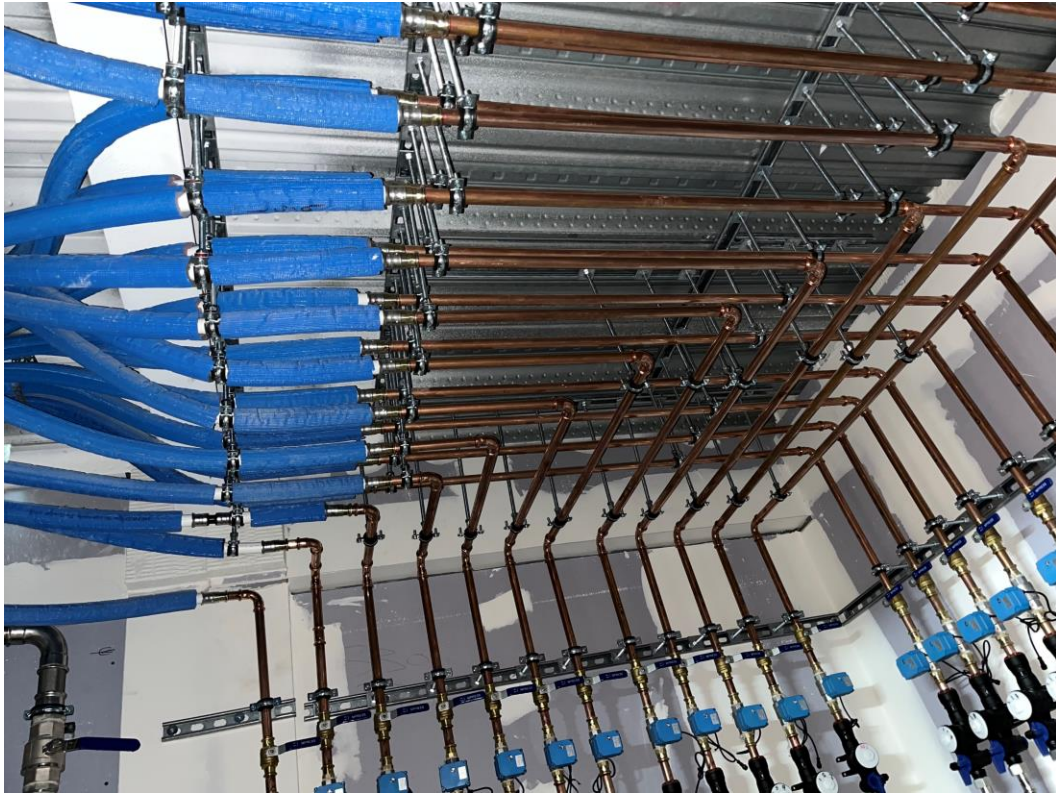
Student Wing – Water meters installed
