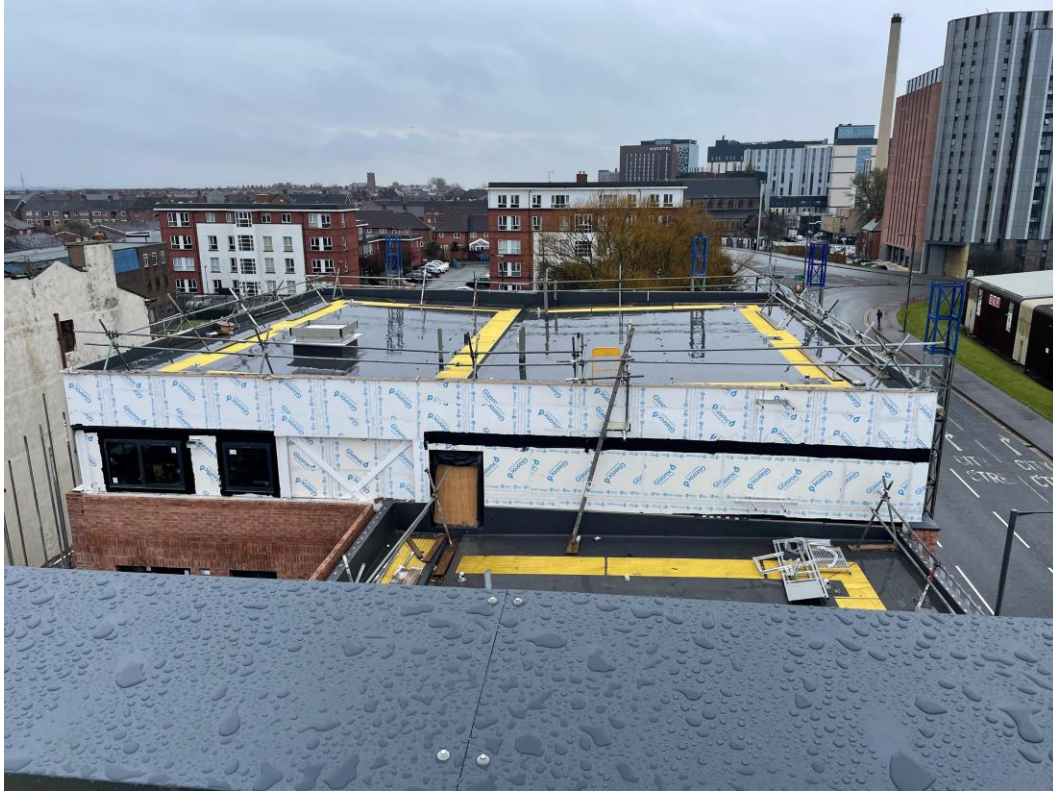
Commercial Block – Weatherboarding installation complete
