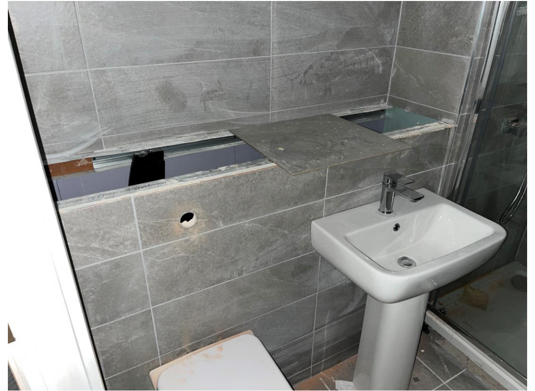
Residential Block – IPS, wall tiling and appliances on-going
