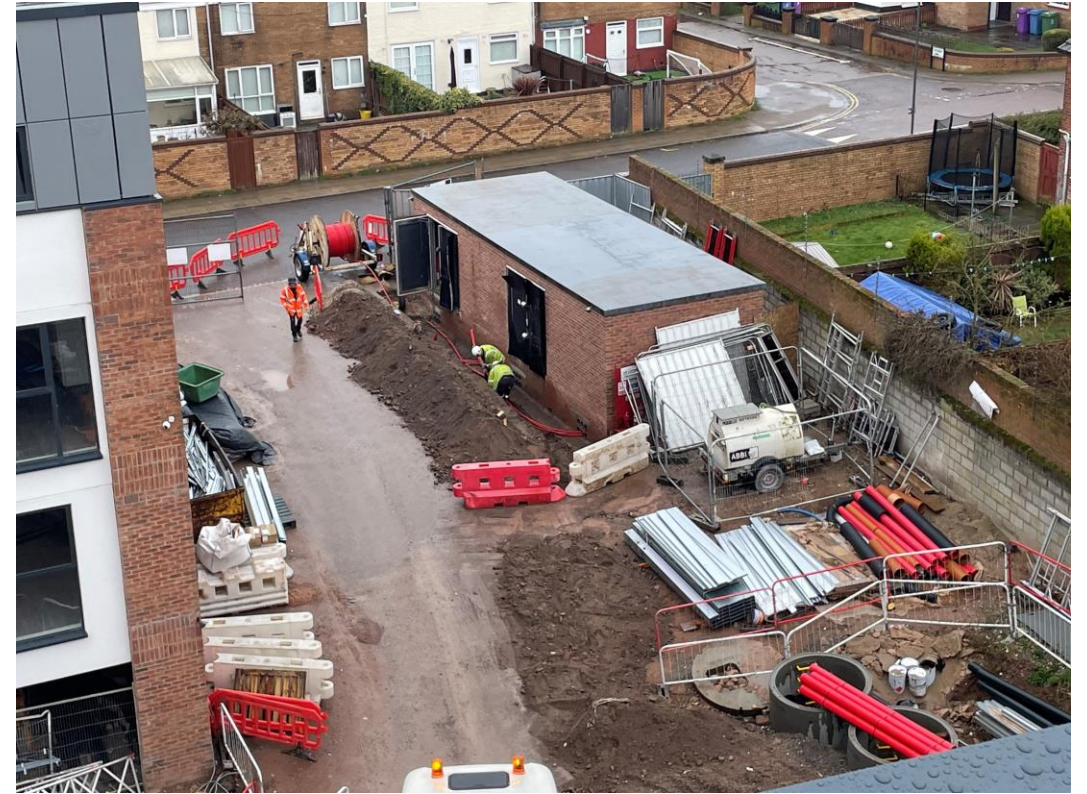
Excavation to substation on-going
