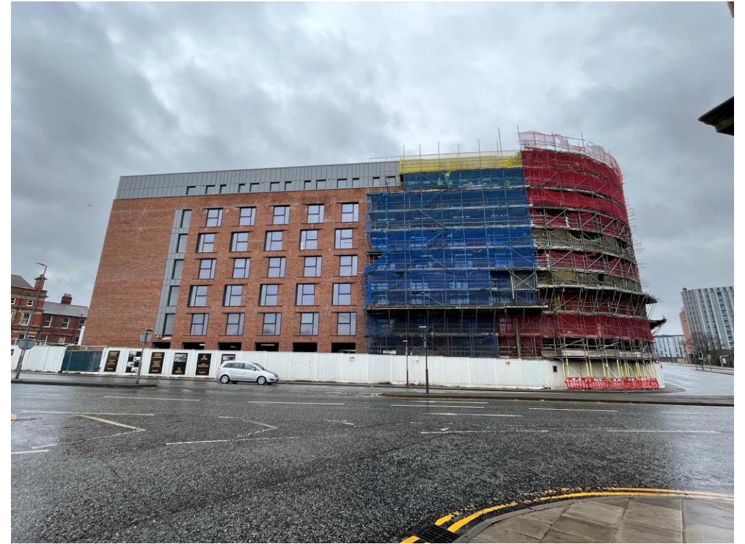
West Derby Road - Site view
