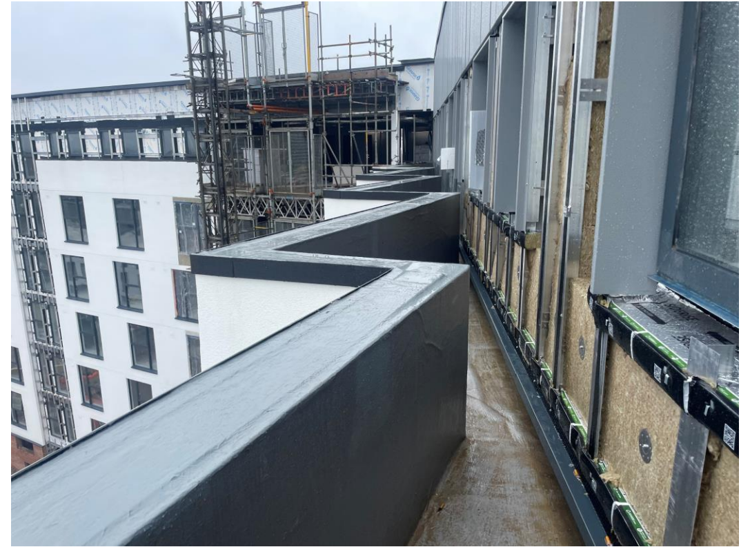
“Zig-zag’ Elevation – Cladding installation on-going
