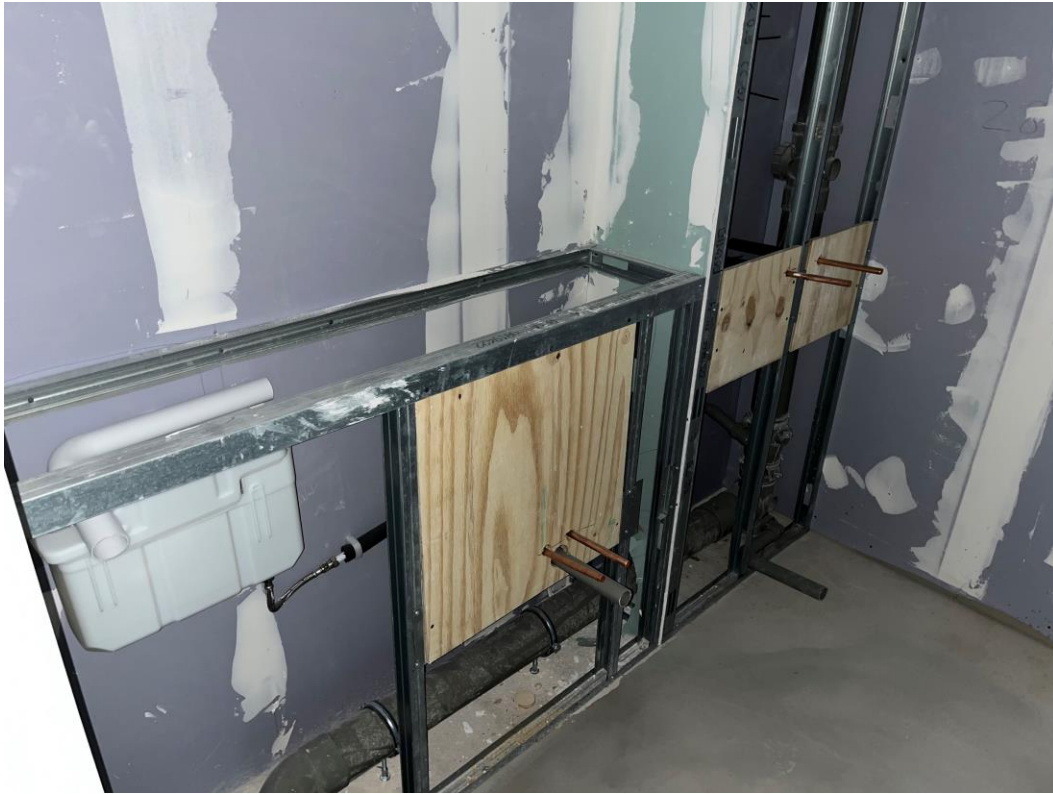
Residential Block – IPS Installed
