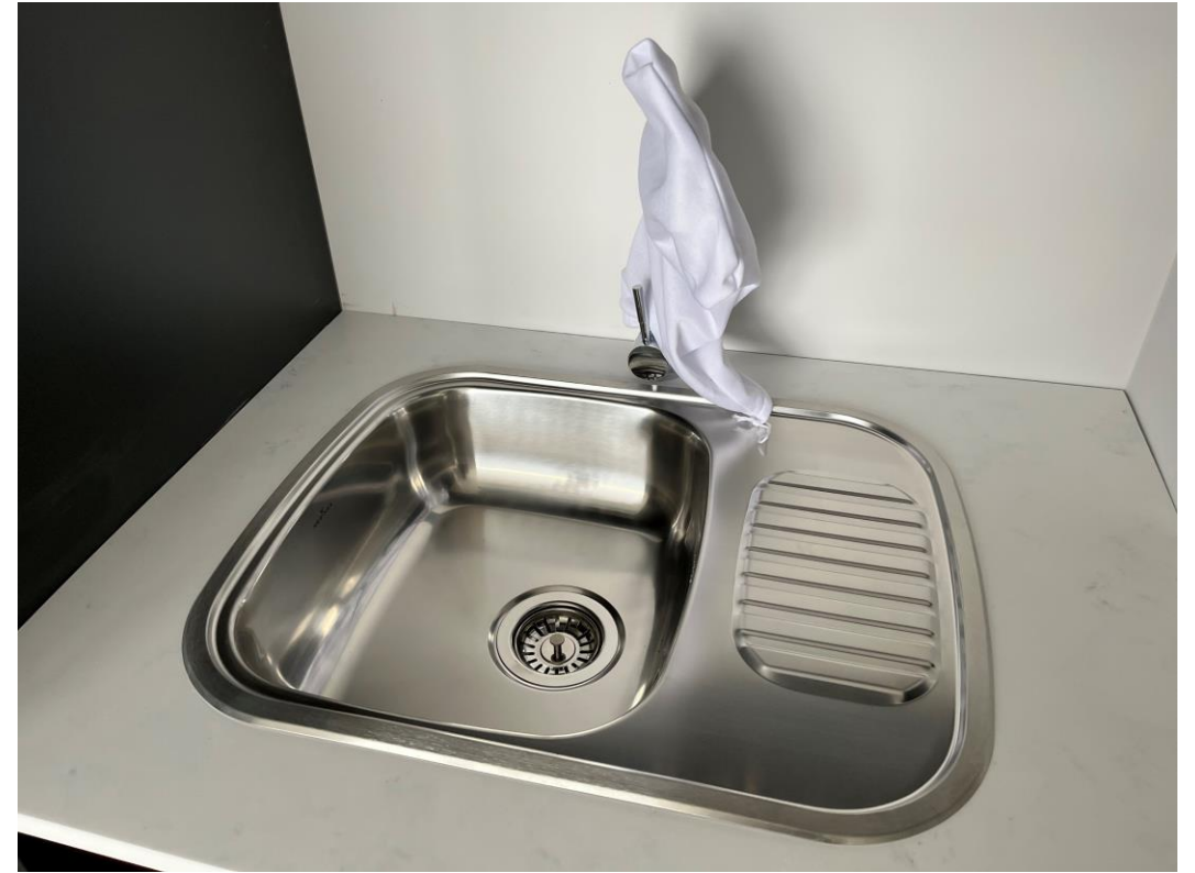
Residential Block – Kitchen sink installation
