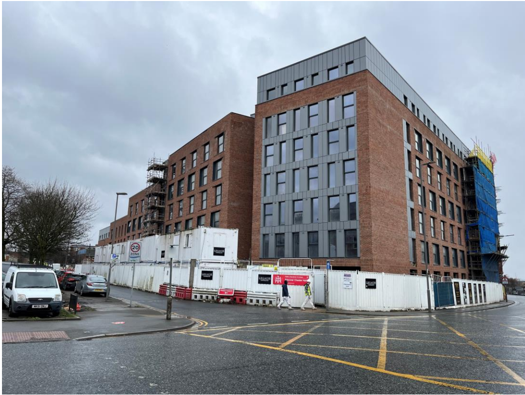
West Derby Road - Site view
