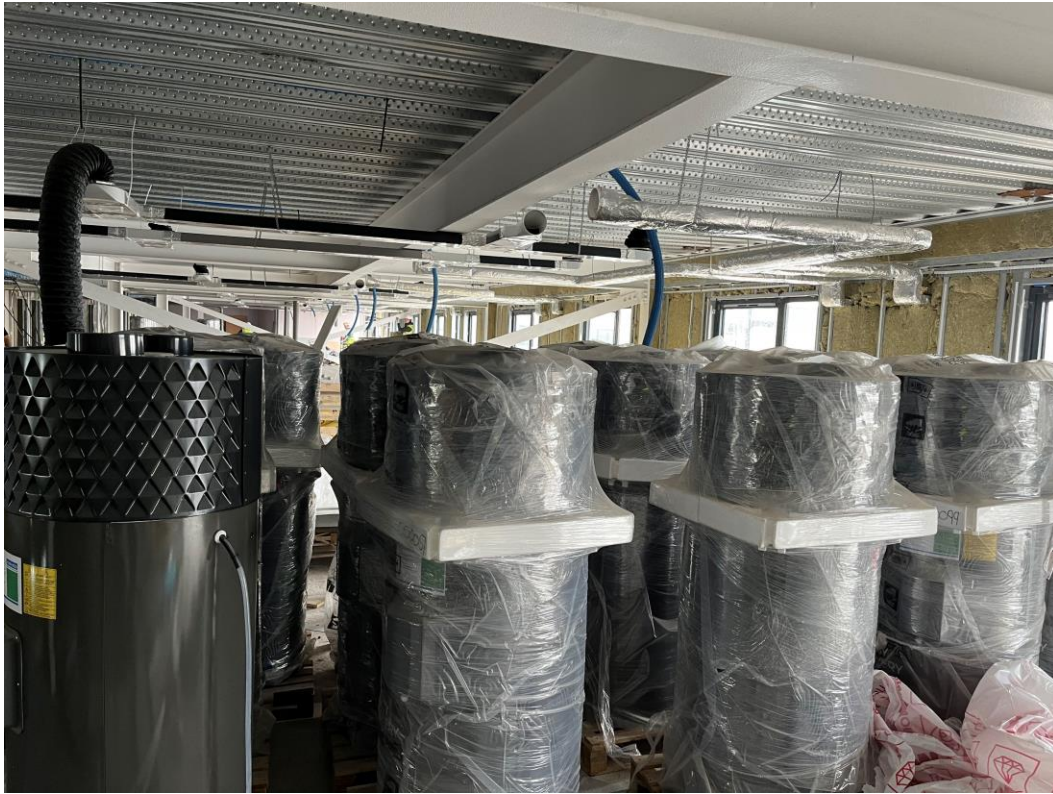
Material storage - KERS units
