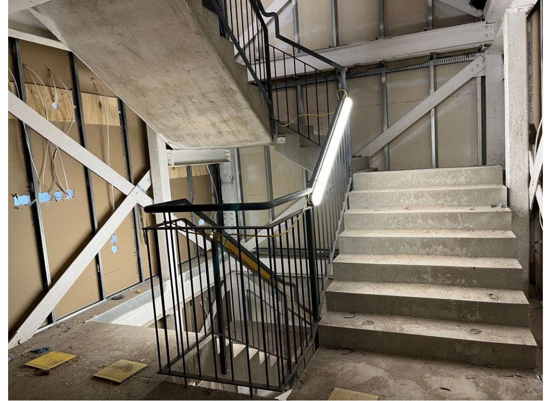
Residential Block – Metal balustrade installation on-going
