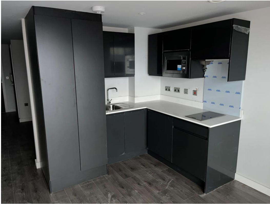
Residential Block – Kitchen complete
