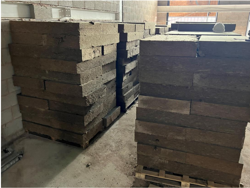
Commercial Wing – Soffit insulation
