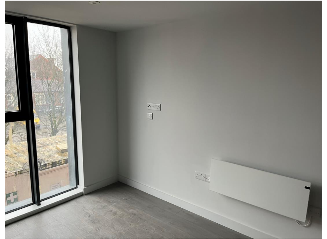
Student Block - Internal finishes on-going
