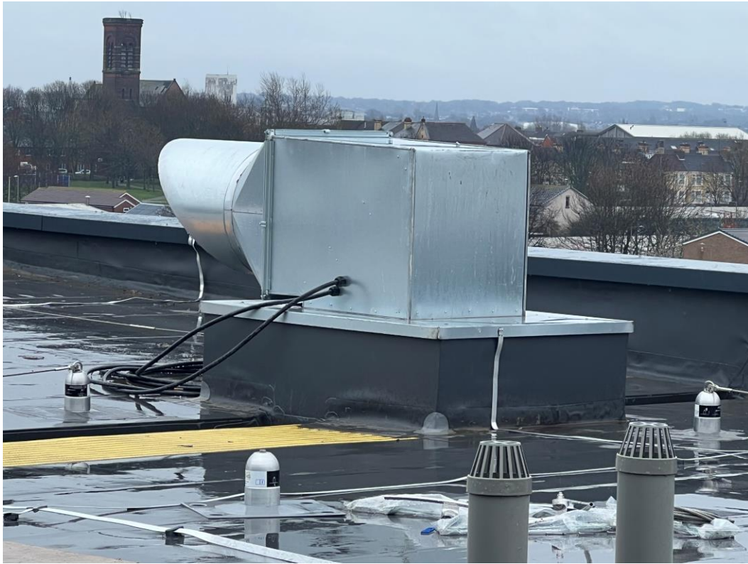
Student Wing – Plant installed to roof
