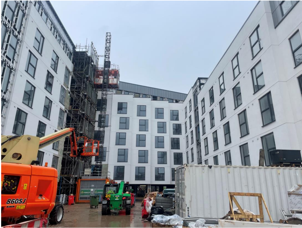
“Zig-zag’ Elevation – Cladding installation on-going
