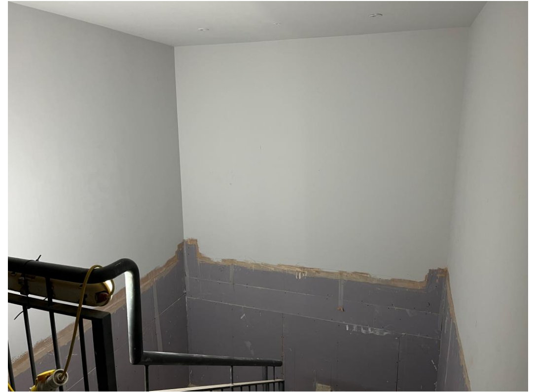
Student Wing – Internal finishes to stairwell on-going
