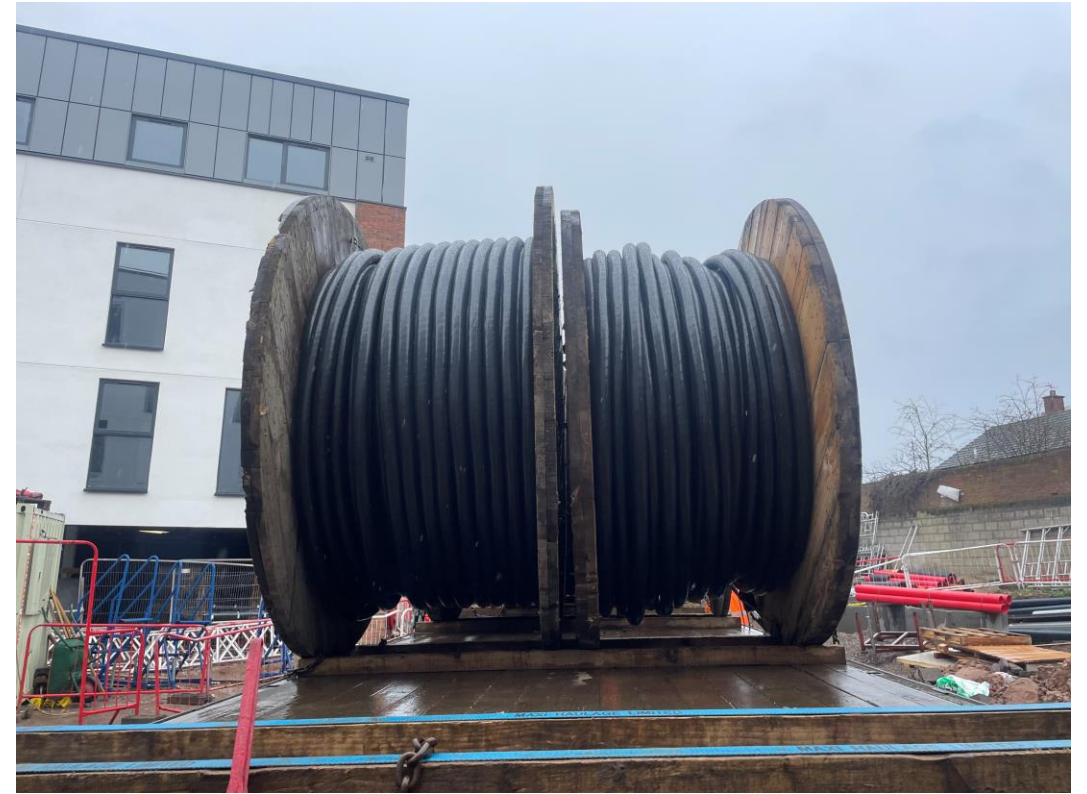
Material Delivery – HV Cable
