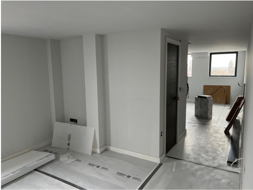
Student Block - Internal finishes on-going
