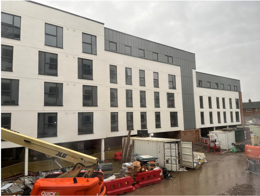
Student Wing – Cladding installation on-going
