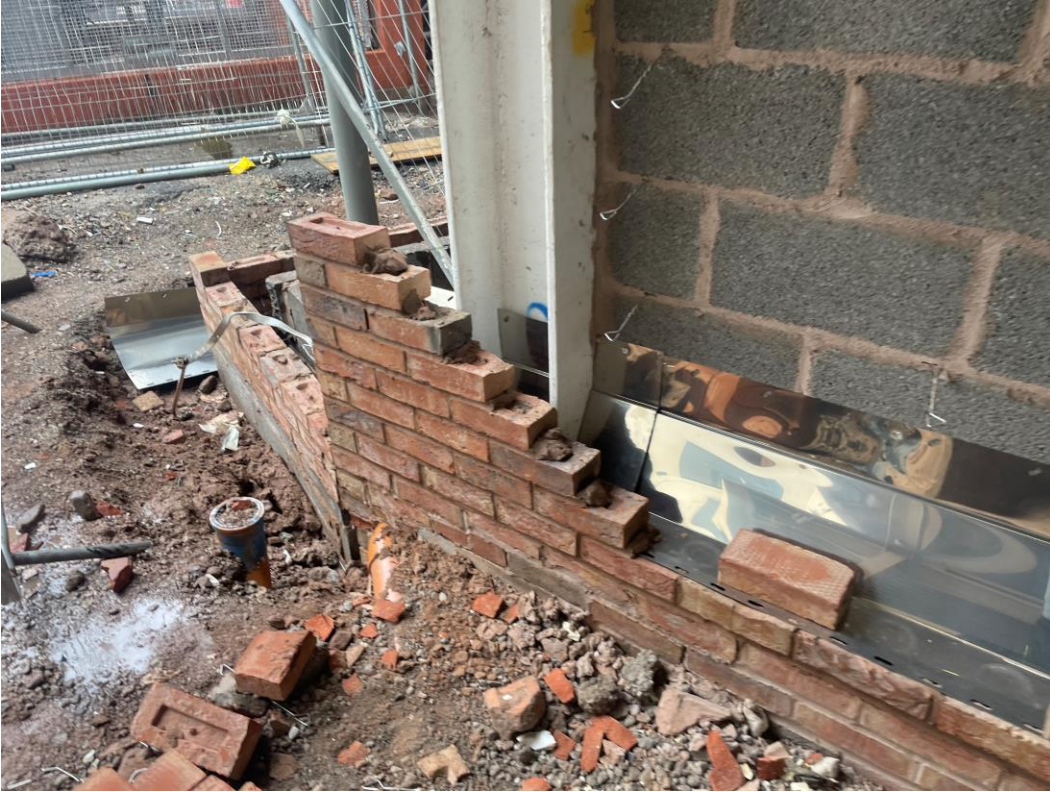
Residential Block - Brickwork installation on-going
