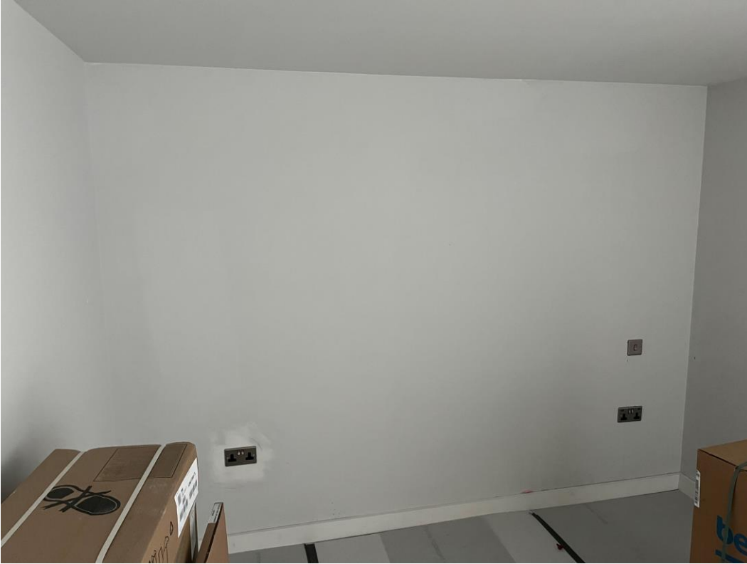
Student Wing – Internal finishes on-going
