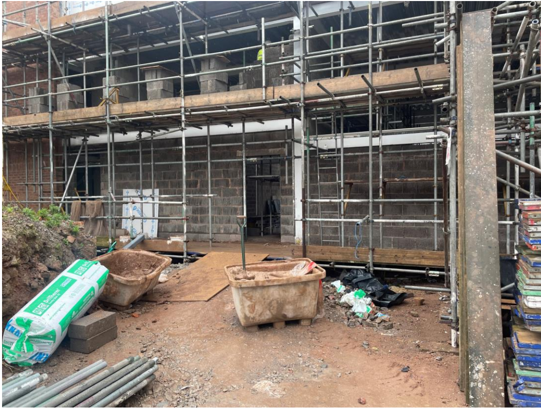
Commercial Block – Scaffolding and External blockwork on-going
