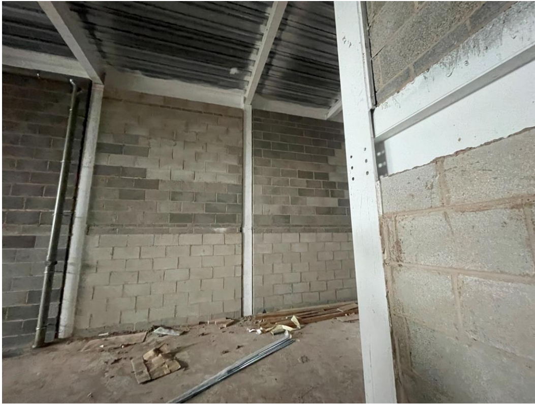
Commercial Block – Internal blockwork on-going
