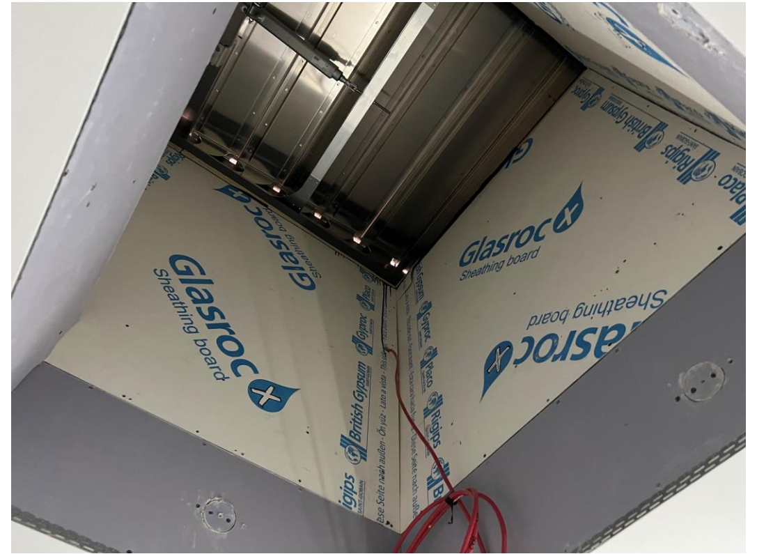
Residential Wing – AOV Installation on-going
