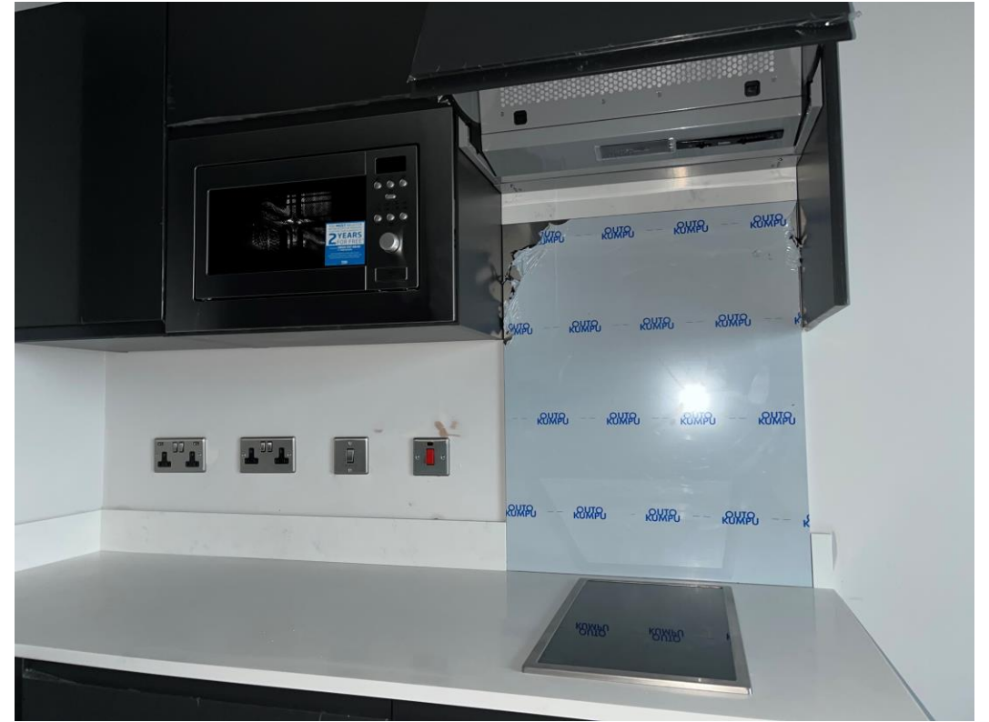
Residential Block – Kitchen appliances installation
