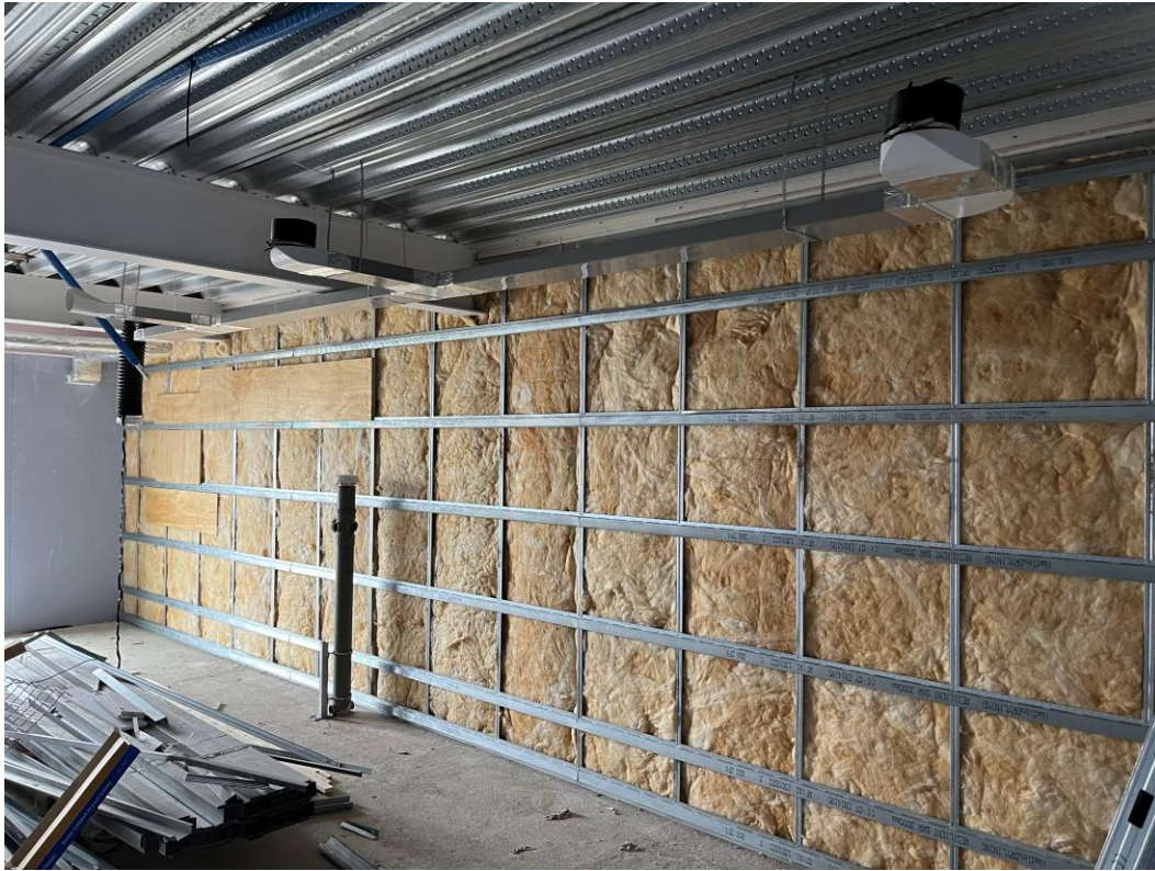
Residential Block – Metal partitions, insulation and pattress installation
