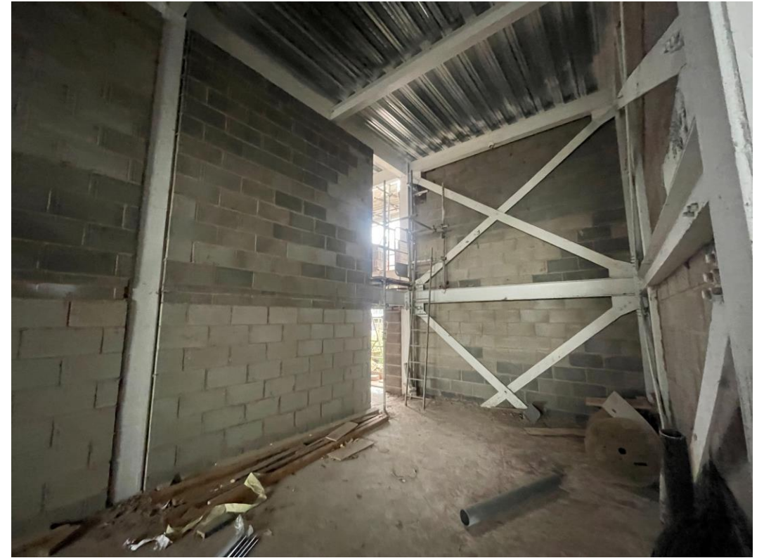
Commercial Block – Internal blockwork on-going
