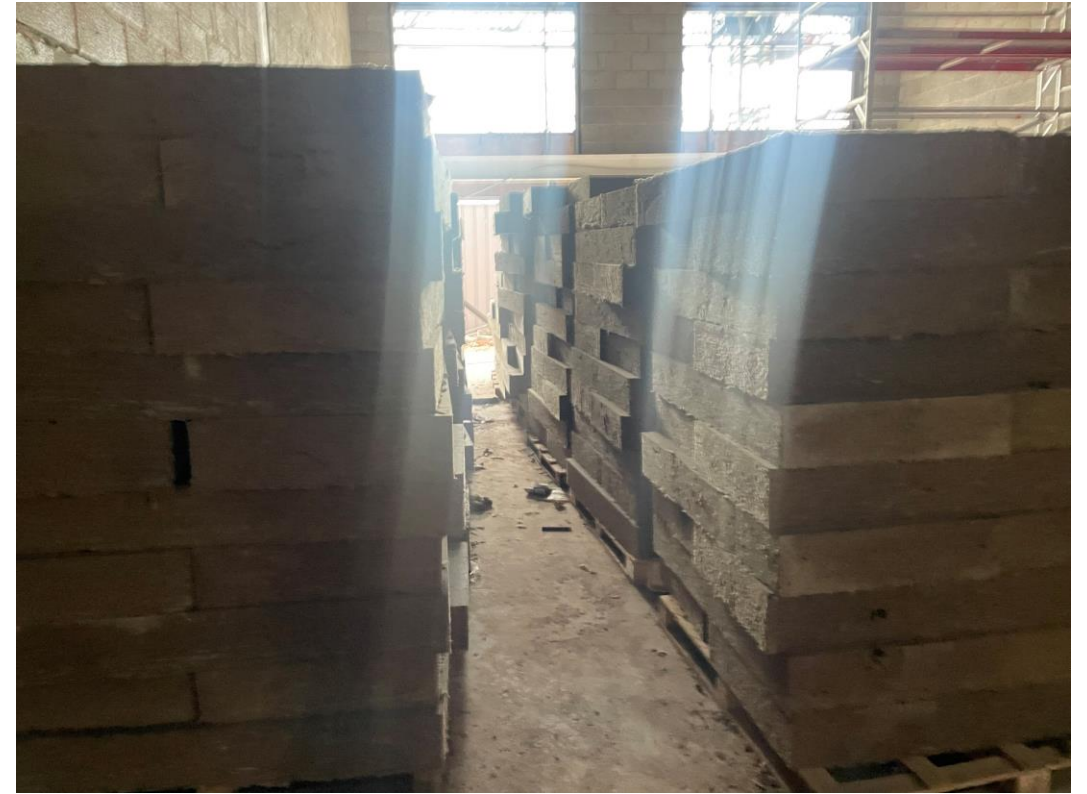
Commercial Wing – Soffit insulation
