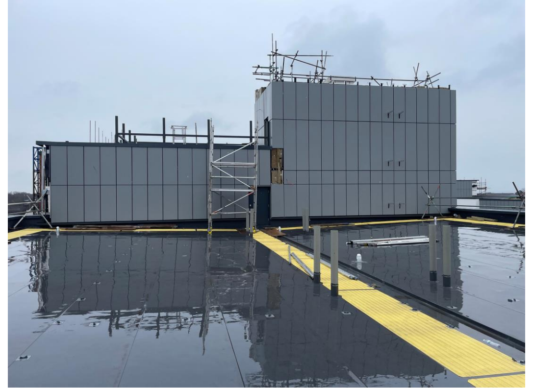
Residential Block – Cladding installation nearing completion
