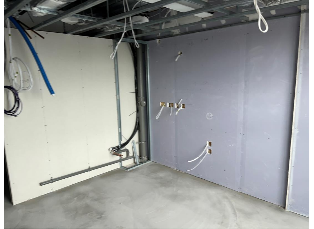
Residential Block – Self-levelling screed on-going
