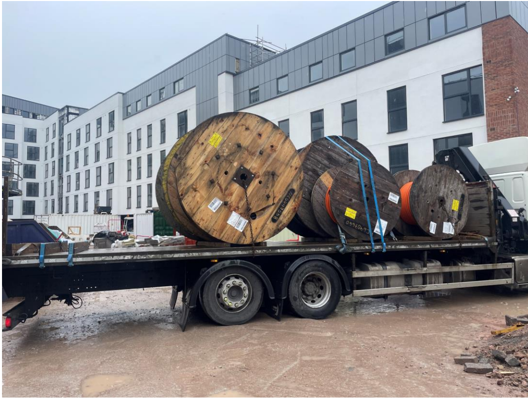
Material Delivery – HV Cable
