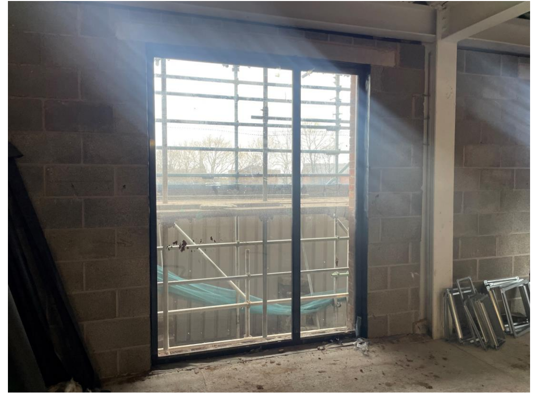
Commercial Block – Window unit installed
