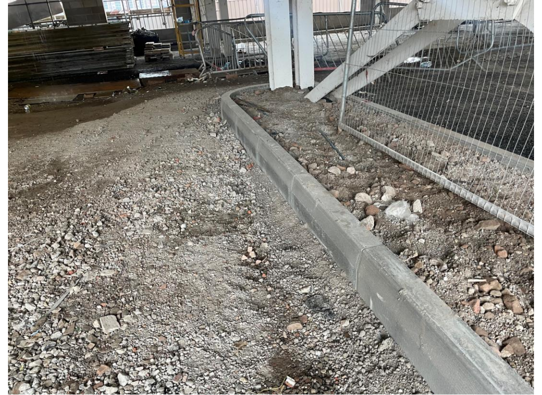
Residential Block - Kerbing installation on-going
