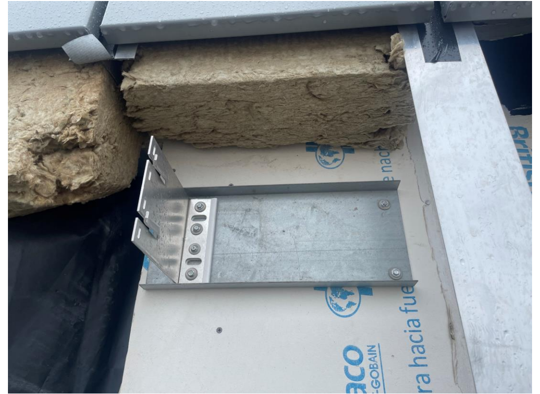
Residential Wing – Cladding rail installation on-going
