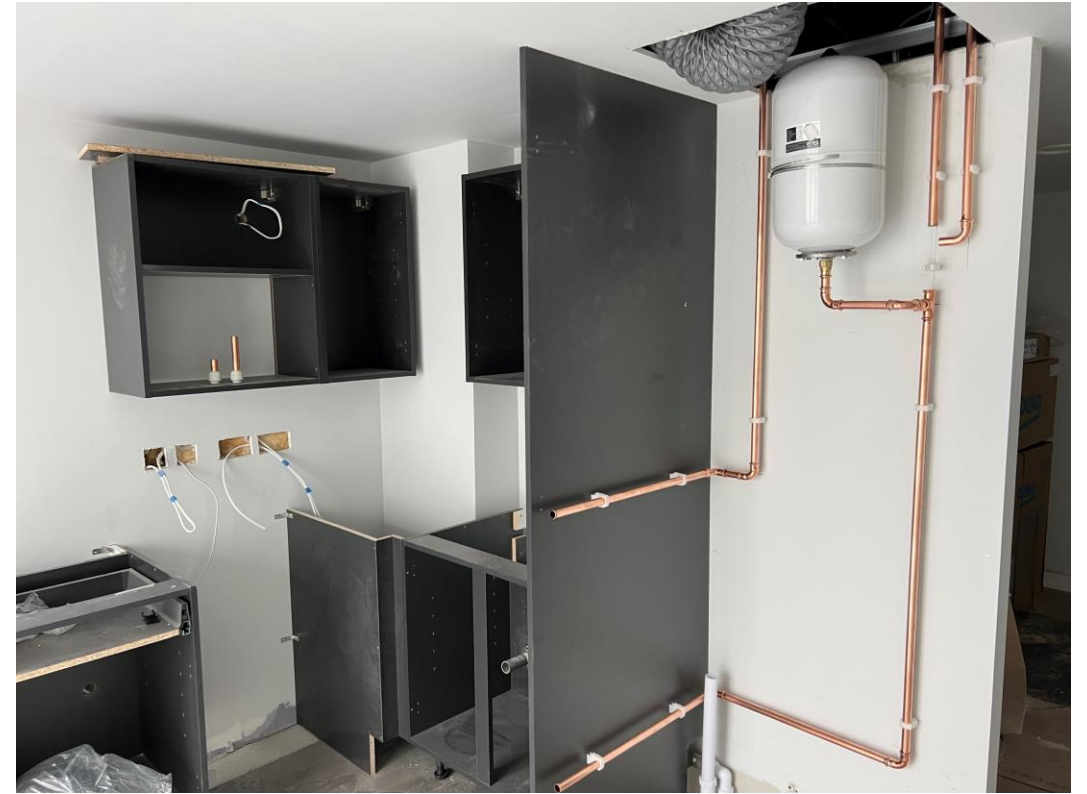
Residential Wing – Kitchen installation
