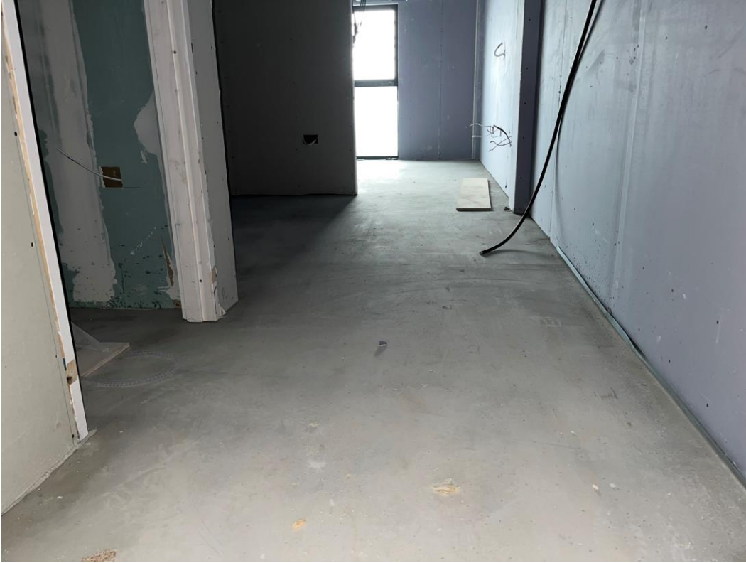
Residential Block – Self-levelling screed on-going
