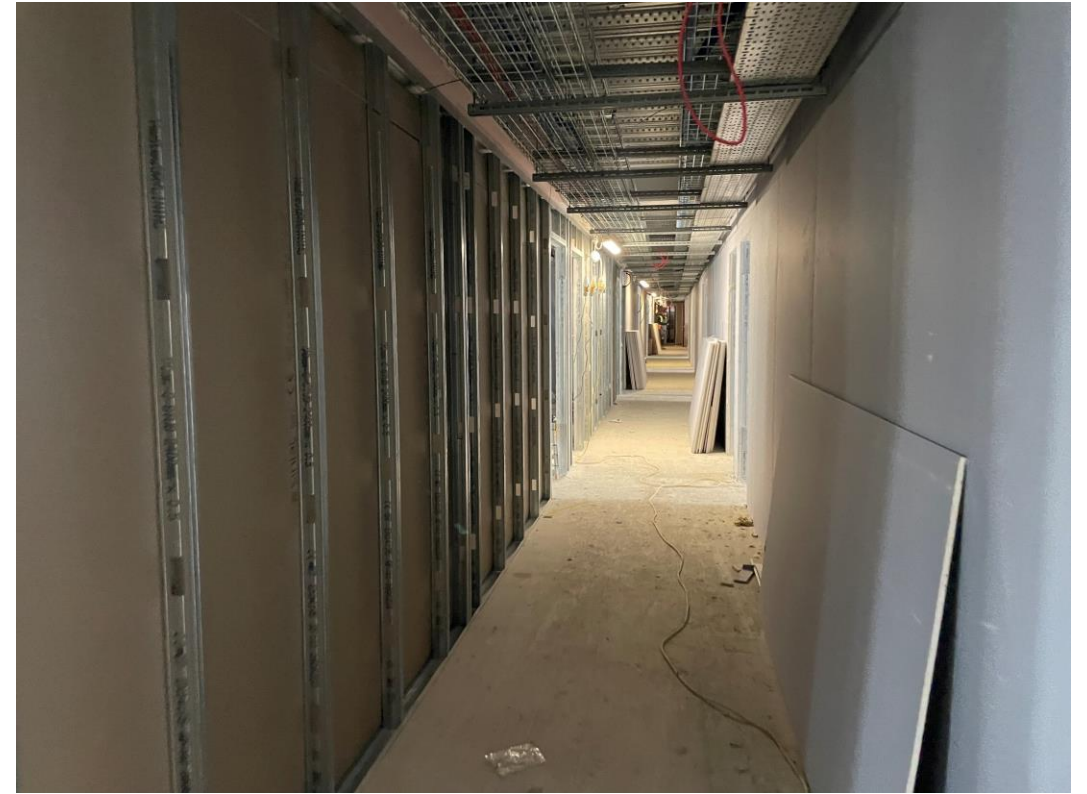
Residential Block – Metal partition erection and boarding
