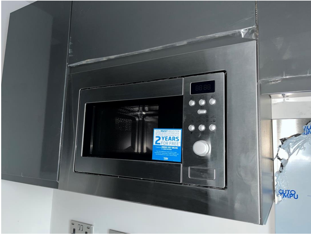
Residential Block – Kitchen appliance installation
