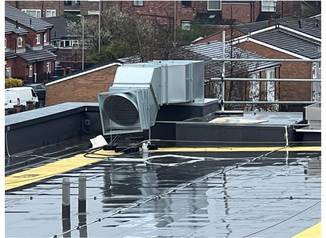
Student Wing – Plant installed to roof
