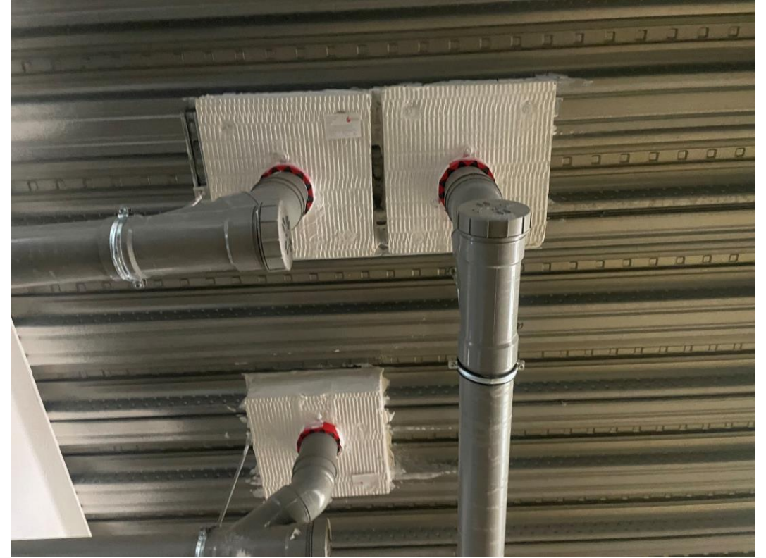
Residential Wing – Fire stopping
