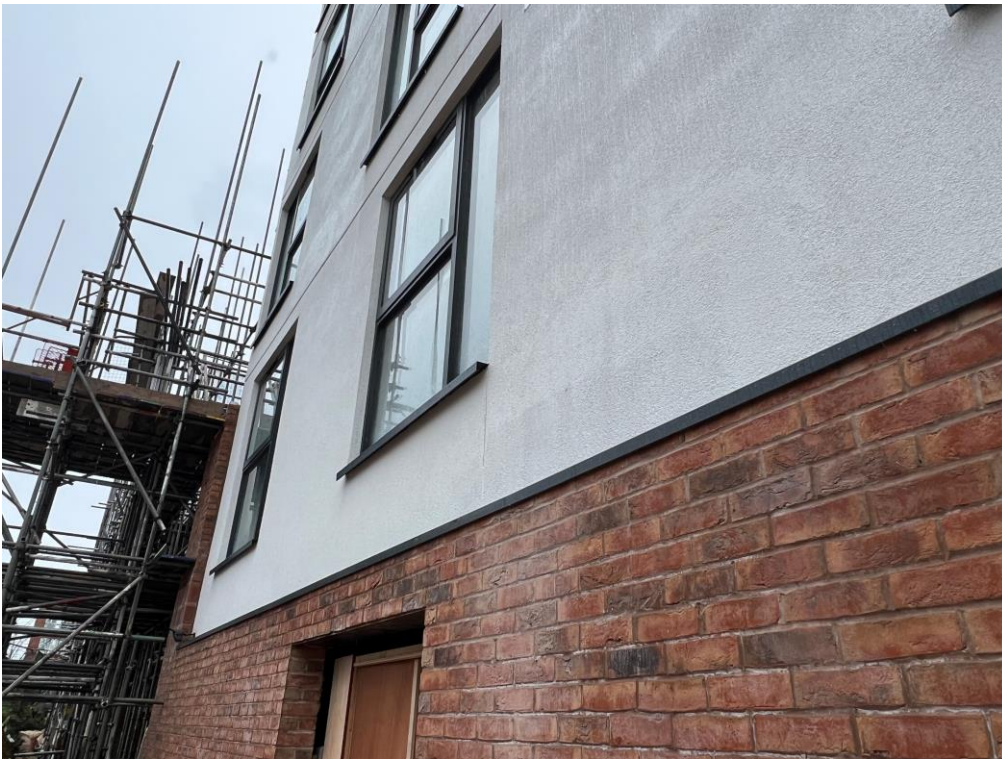
Capping installed to brickwork
