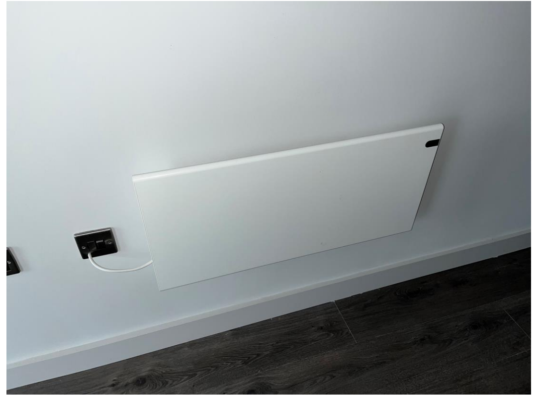
Residential Block – Radiator installation
