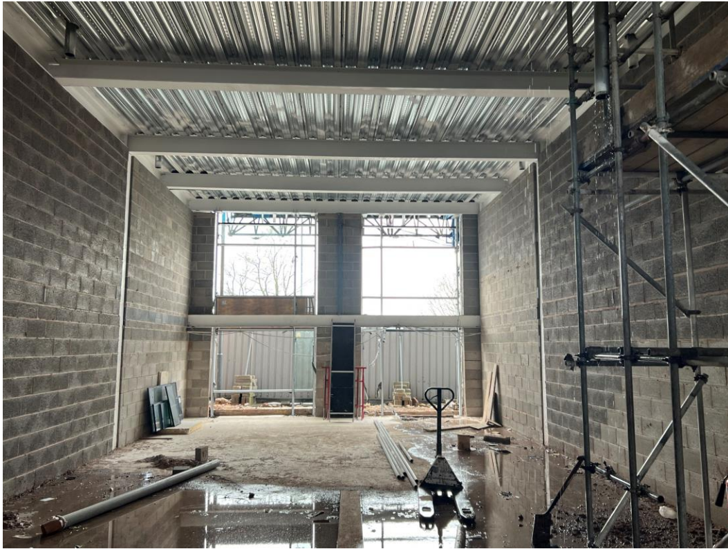
Commercial Block – Curtain walling installation on-going
