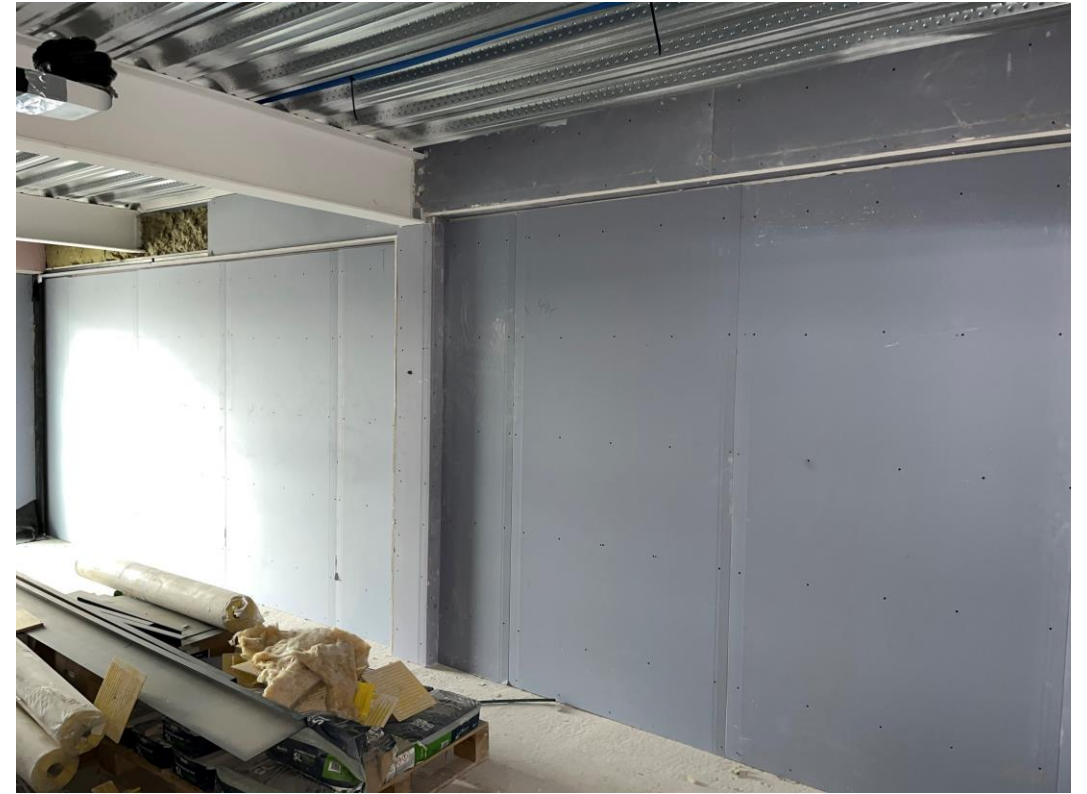
Residential Block – Boarding of partition walls
