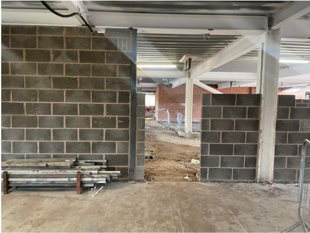
Residential Block – Internal blockwork on-going
