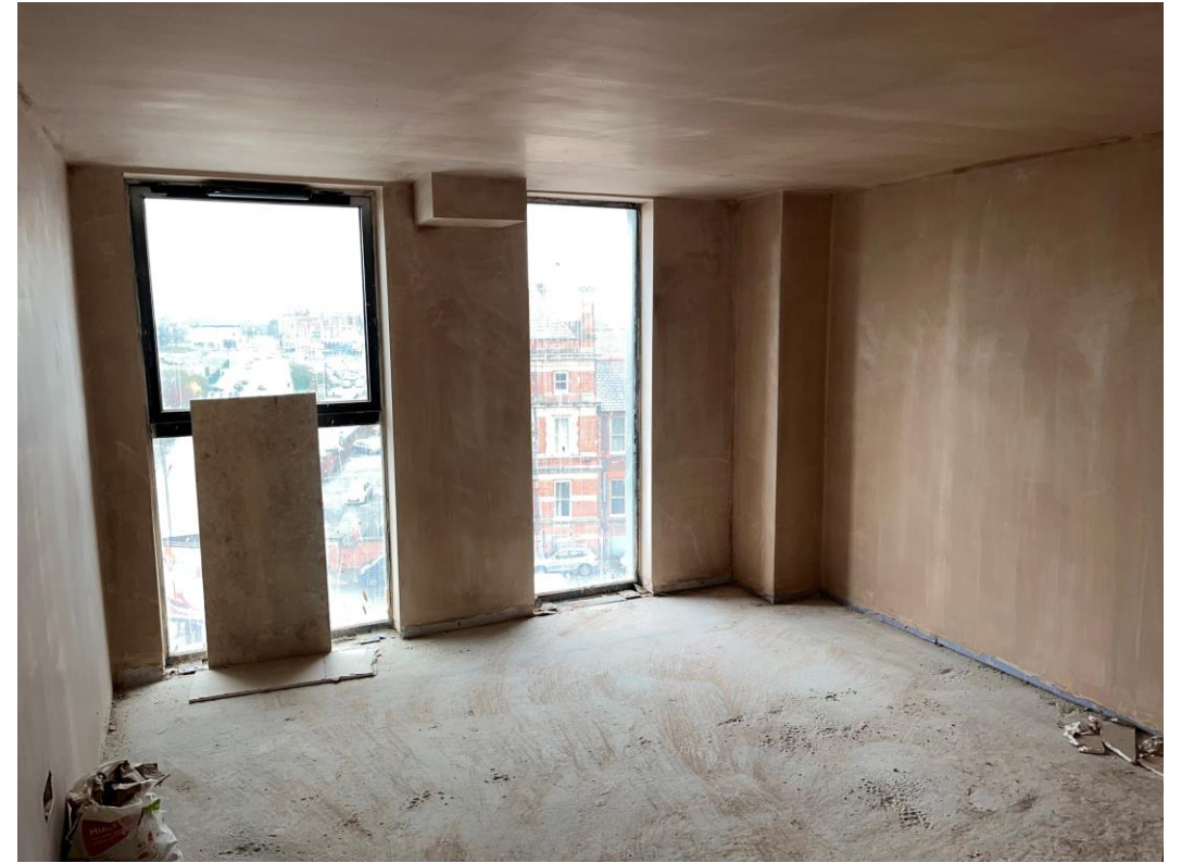
Student Block – Plastering on-going
