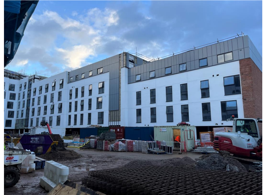
Student wing – Cladding installation ongoing
