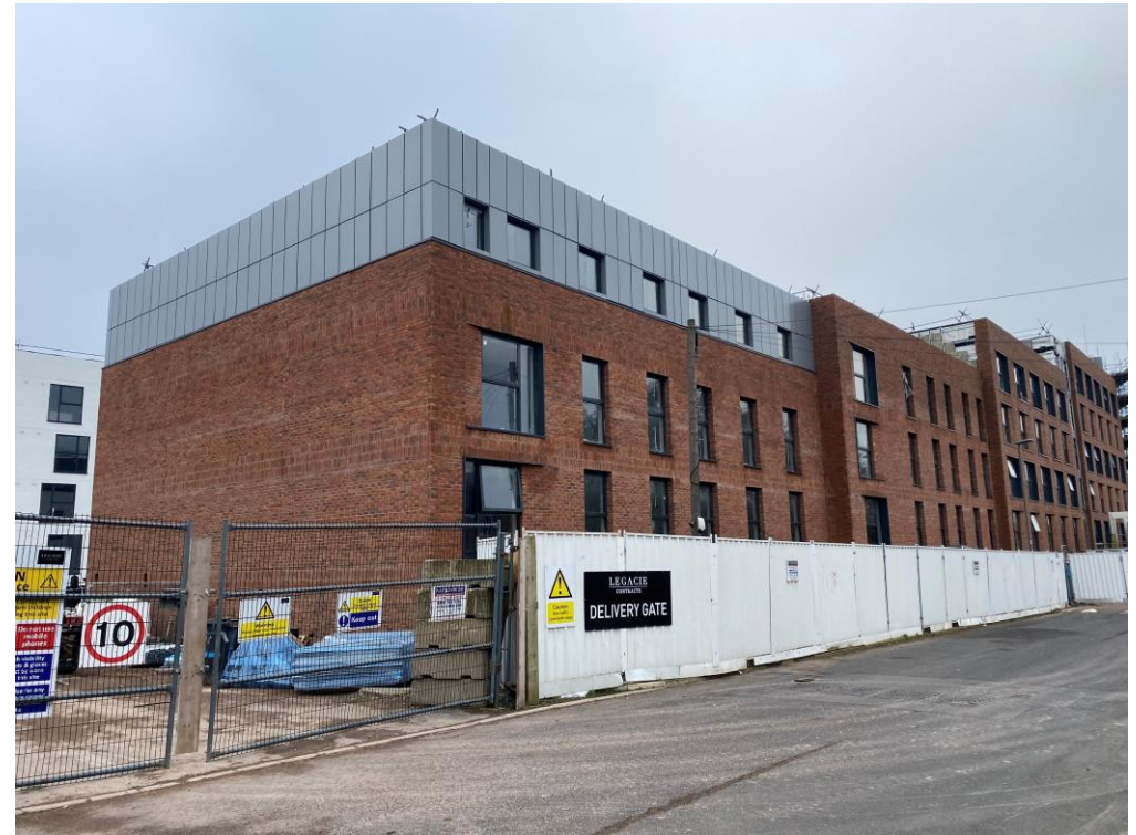
Walker Street - Site view
