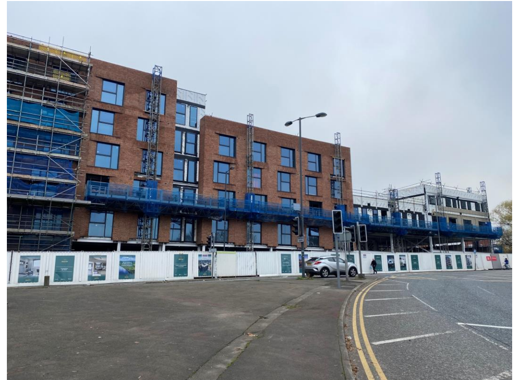
Brunswick Road - Site view
