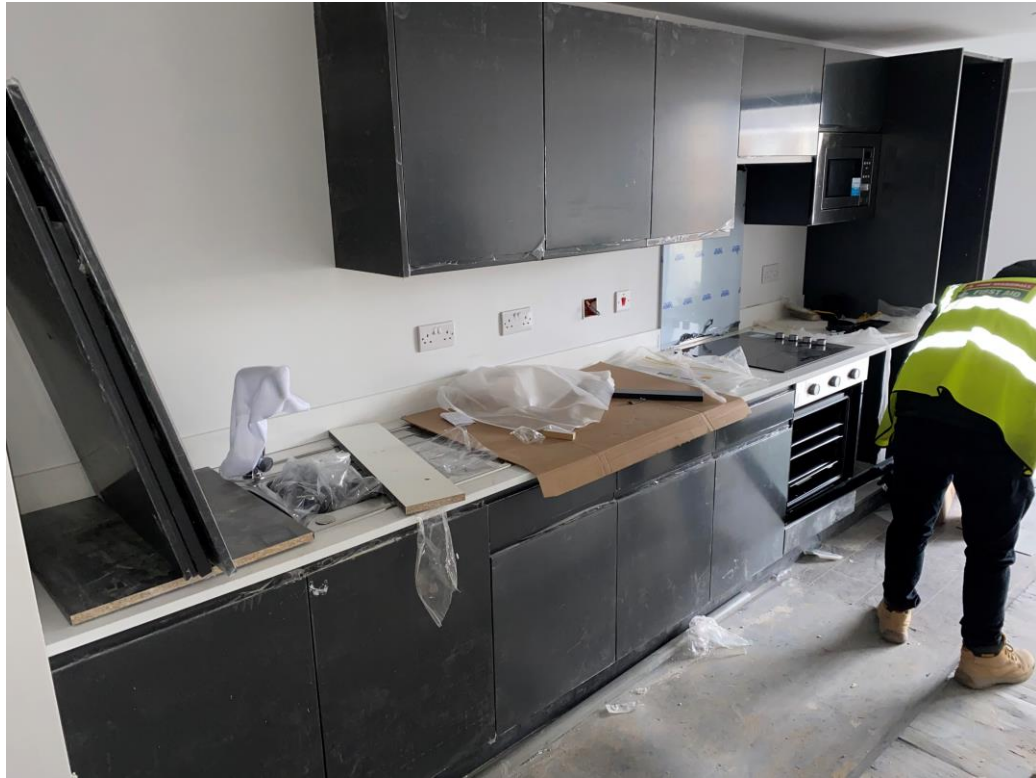
Student Wing – Kitchen ongoing
