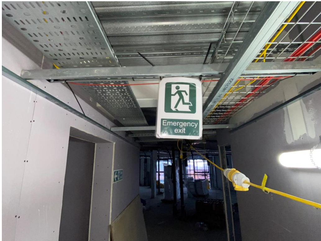
Student Wing – Fire exit signage
