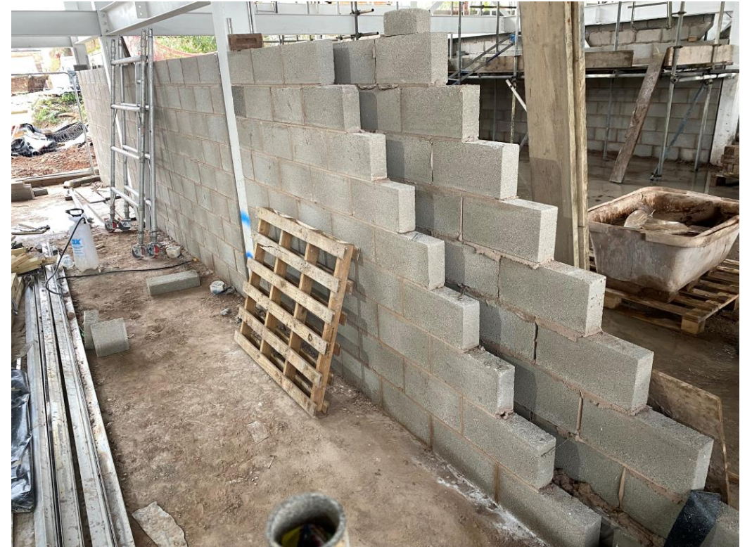
Commercial Units – Internal blockwork cavity wall ongoing
