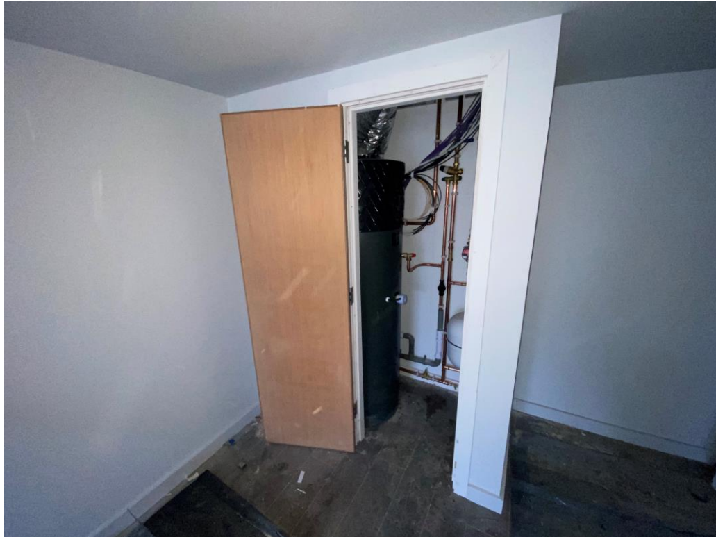
Student Wing – KERS united and internal door installation
