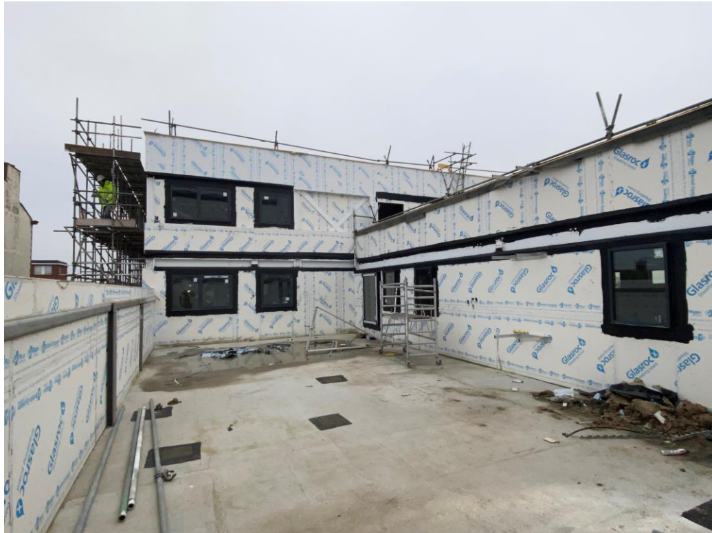
Commercial Block – Weatherboarding on-going
