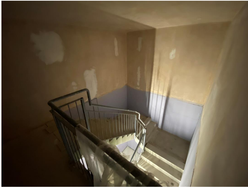
Student Wing – stairwell enclosure
