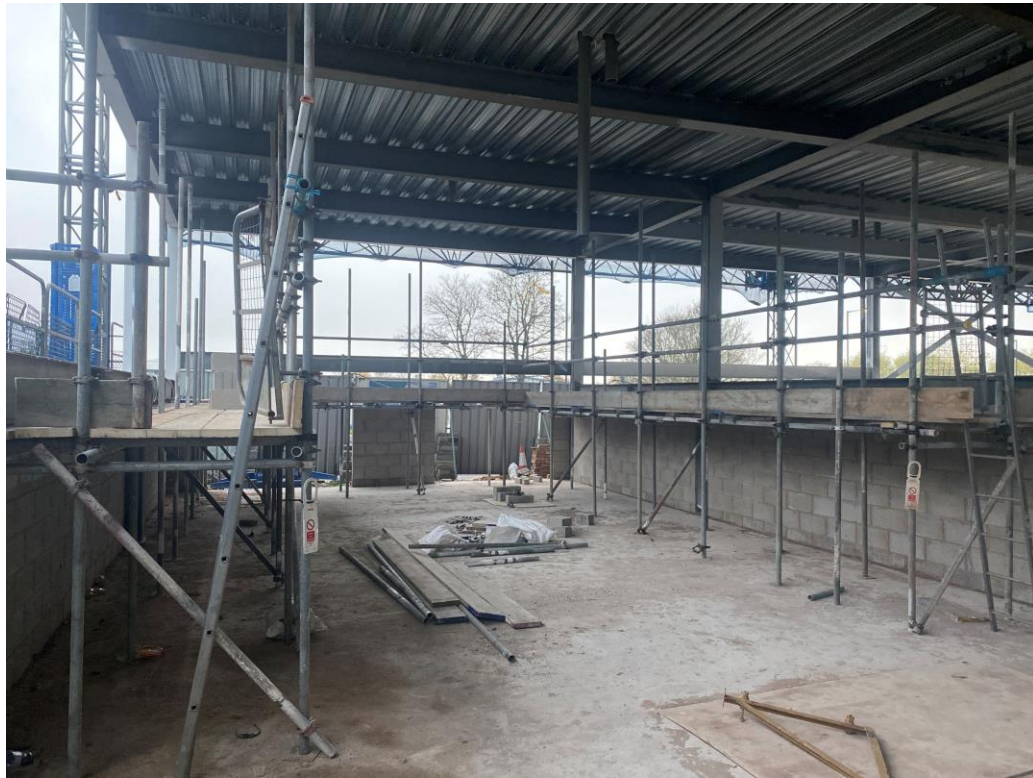
Commercial Units – Blockwork ongoing
