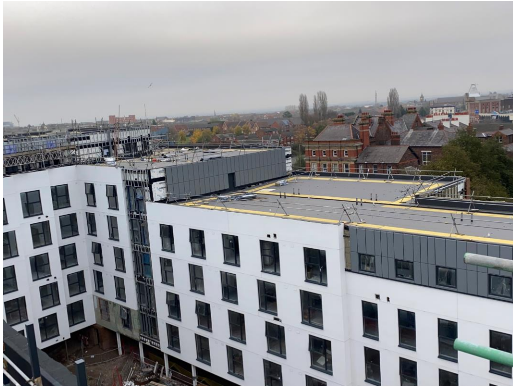
Student Wing – Roof works and cladding ongoing
