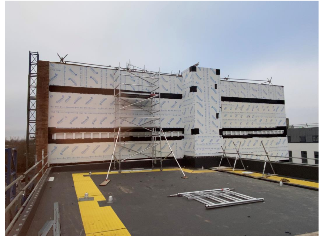
Residential Wing – Weatherboard installation ongoing
