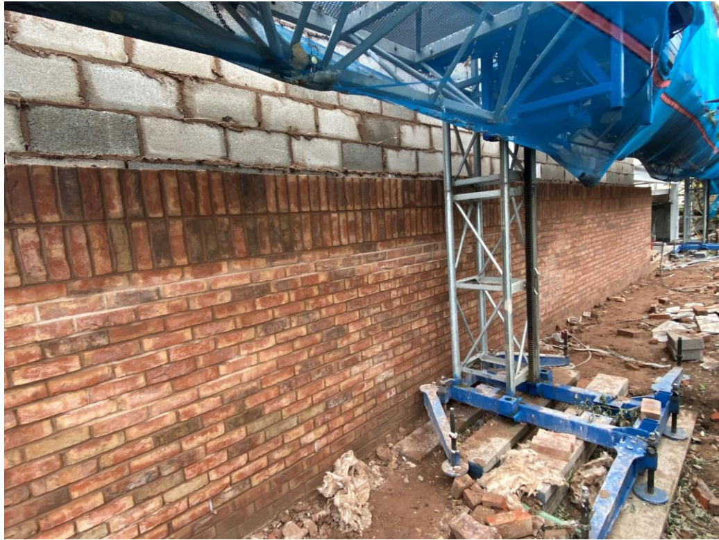
Residential Wing – External brickwork ongoing
