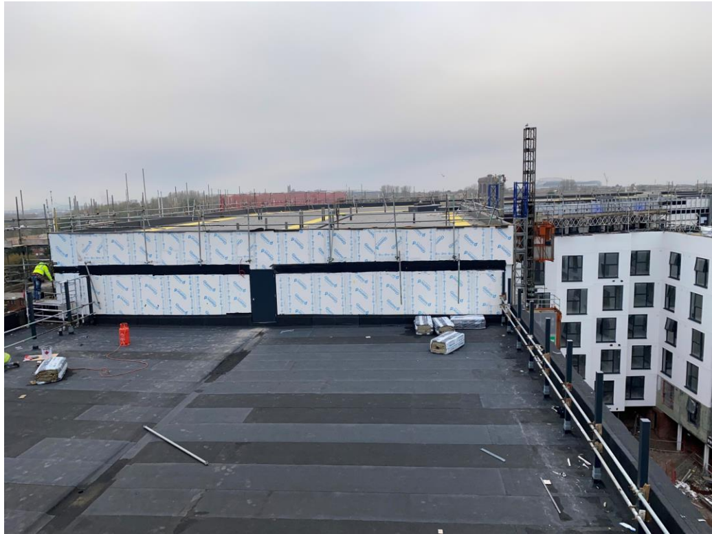
Residential Wing – Weatherboarding and edge protection
