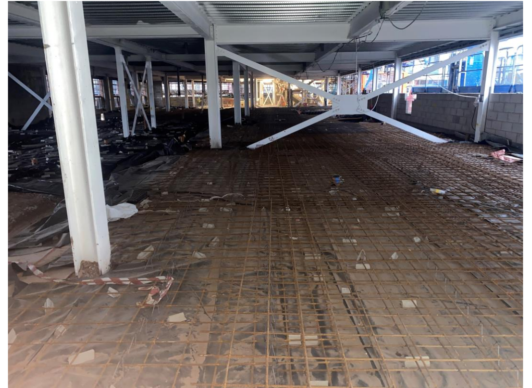
Residential Wing – Ground floor slab preparation and rebar installation
