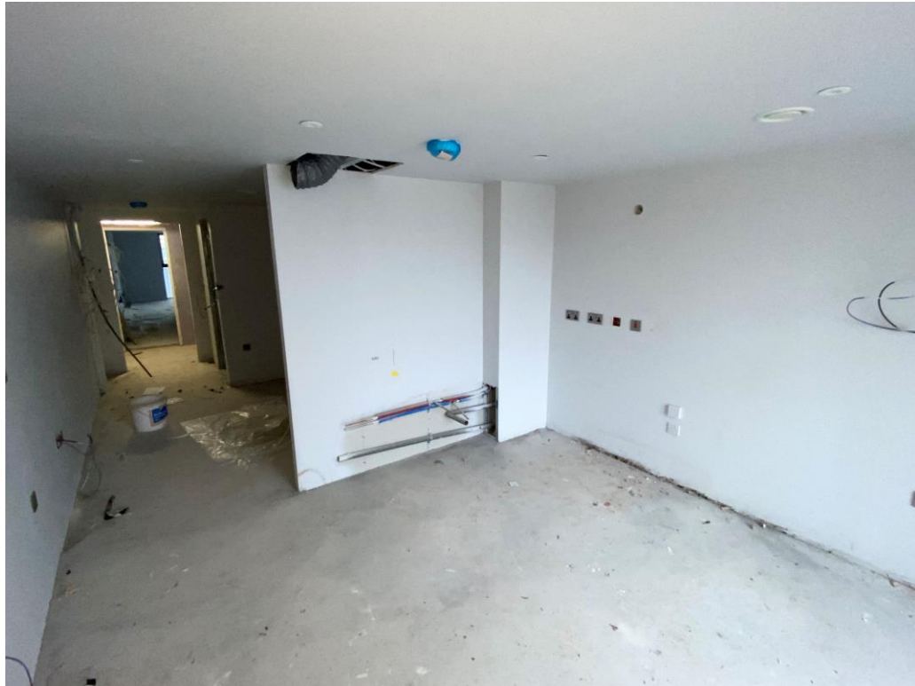
Residential Wing – Screed and Internal finishes on-going
