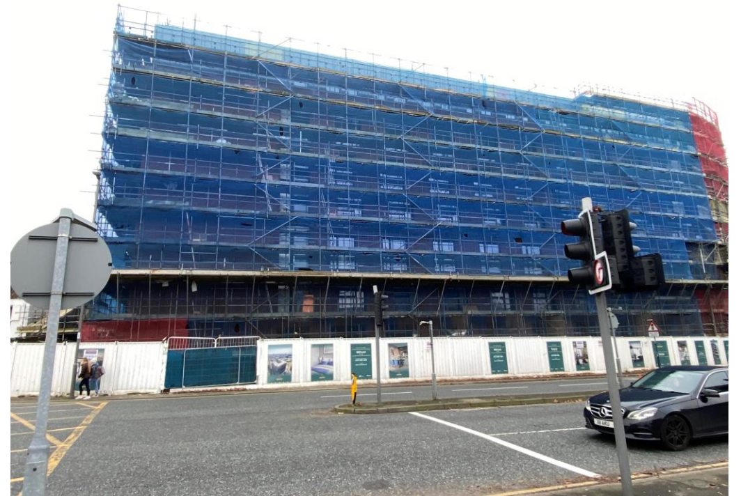
West Derby Road - Site view
