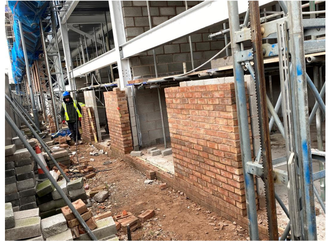
Residential Wing – External brickwork progress
