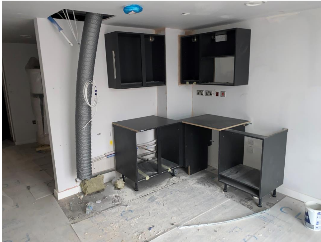
Residential Wing – Kitchen on-going
