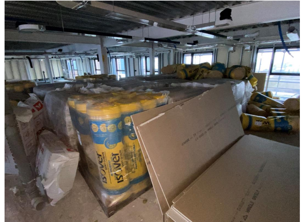
Material storage – Insulation Roll
