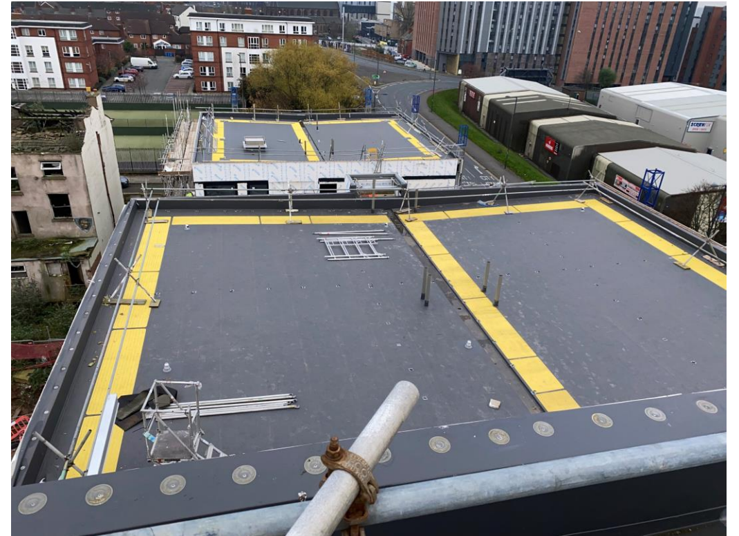
Commercial Block – Mansafe, weatherboarding and edge protection
