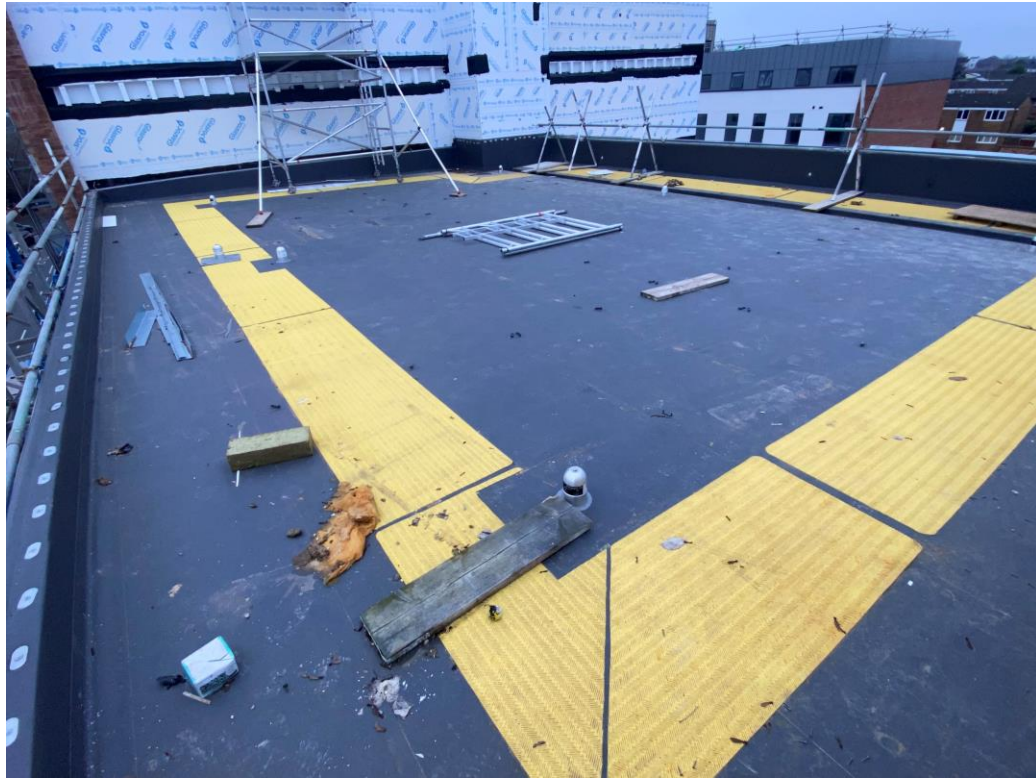
Residential Wing – Weatherboard installation ongoing
