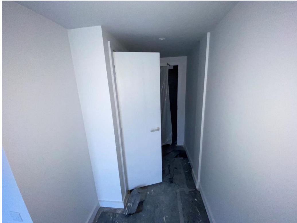
Student Wing – Internal finishes ongoing
