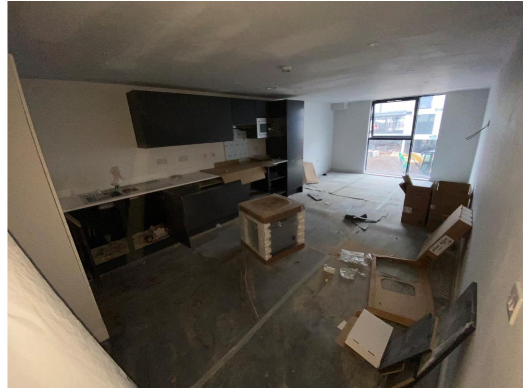
Student Wing – kitchen and living area ongoing
