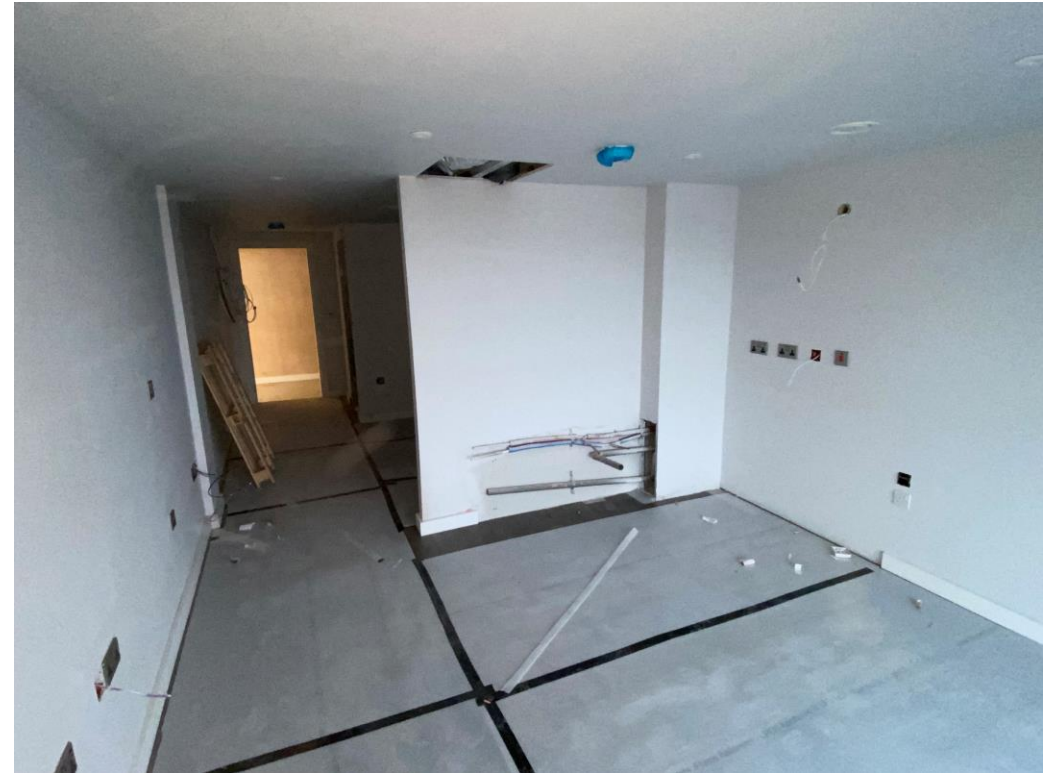
Residential Wing – Laminate flooring and Internal finishes on-going
