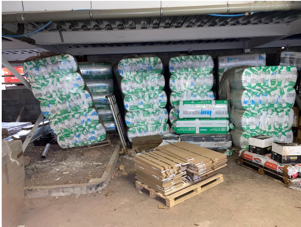
Material Storage – Rocksil Insulation
