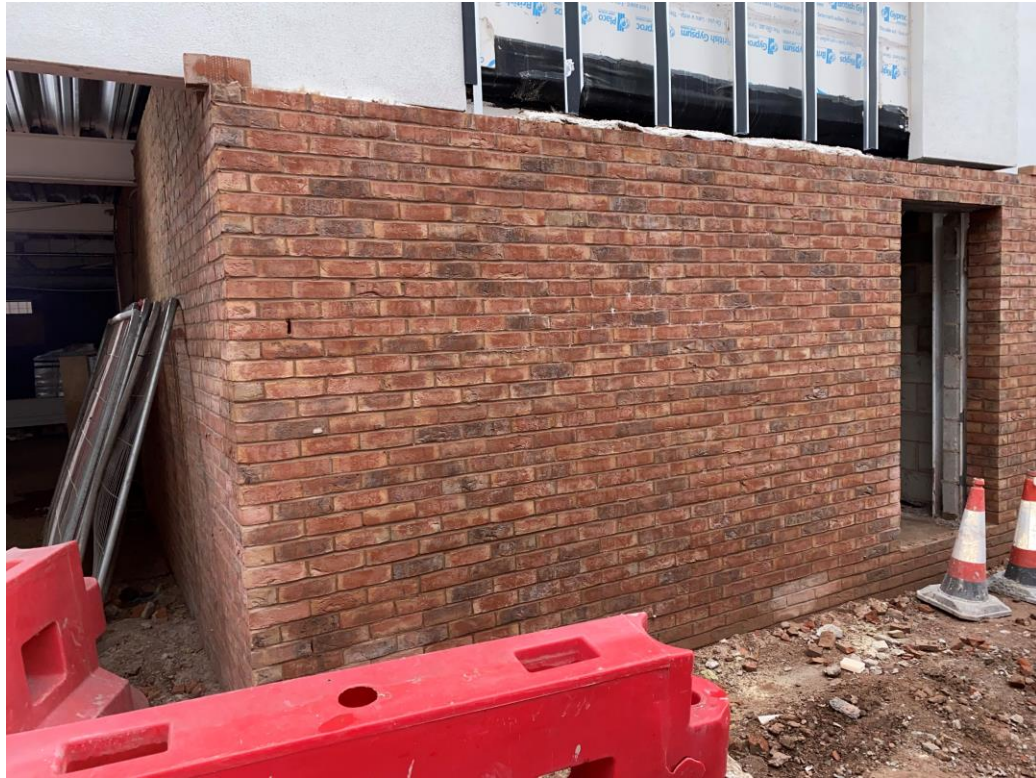
Student Wing – External brickwork ongoing
