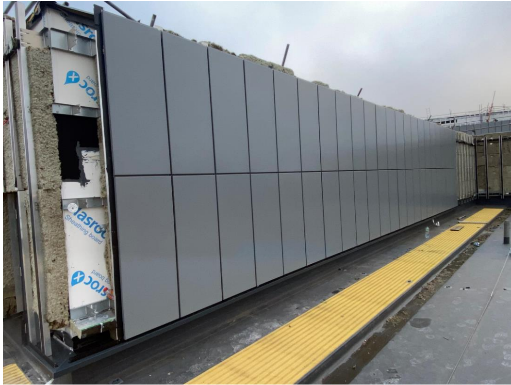
Student Wing – External insulation and cladding on-going
