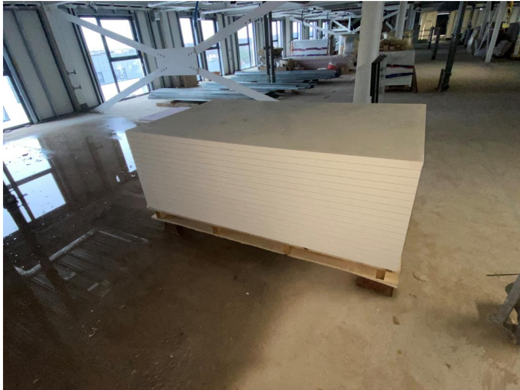
Material storage wall linings
