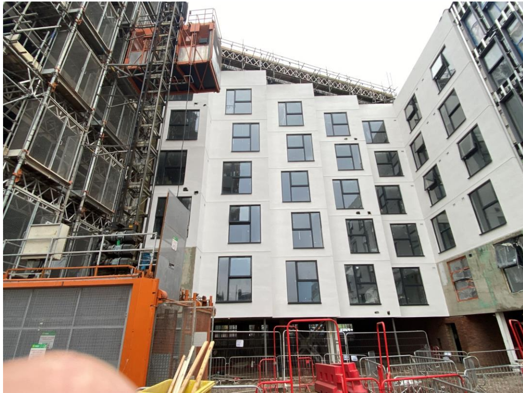
'Zig-zag' Elevation – Render & render coat decoration
