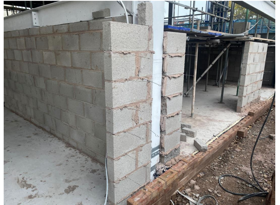
Commercial Units – Blockwork and brickwork ongoing
