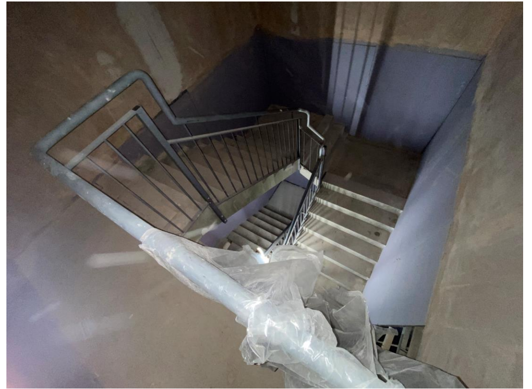
Student Wing – stairwell enclosure
