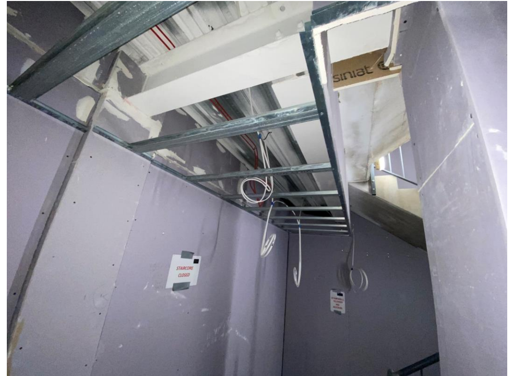
Residential Wing – Ceiling grid and 1 st fix electrical installation
