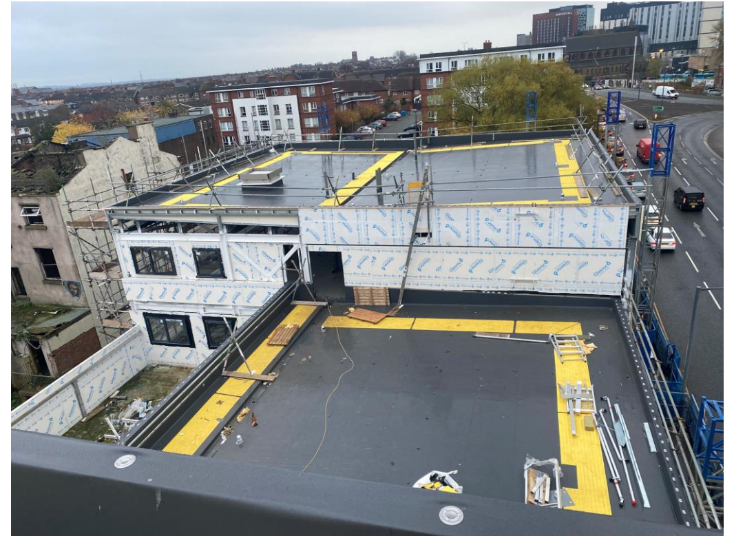
Commercial Block – Weatherboarding and roof works ongoing
