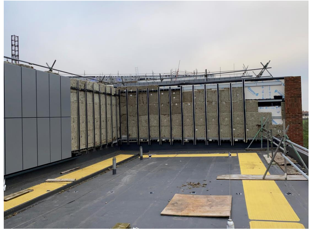
Student Wing – External insulation and cladding on-going
