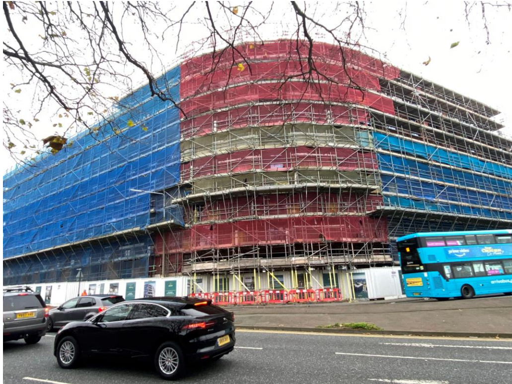
Brunswick Road - Site view
