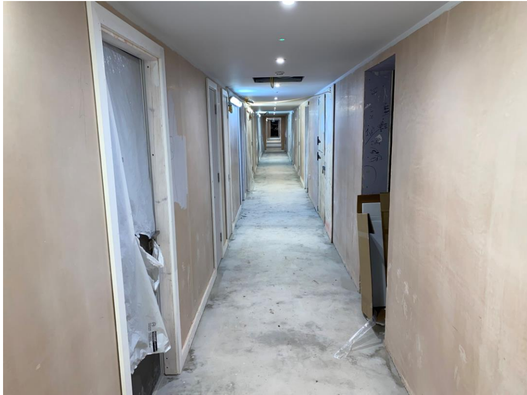
Student Wing – Internal finishes on-going
