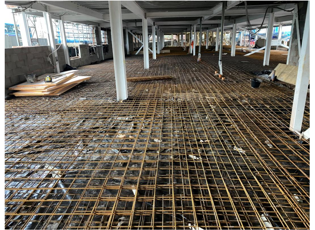
Residential Wing – Ground floor slab rebar installation
