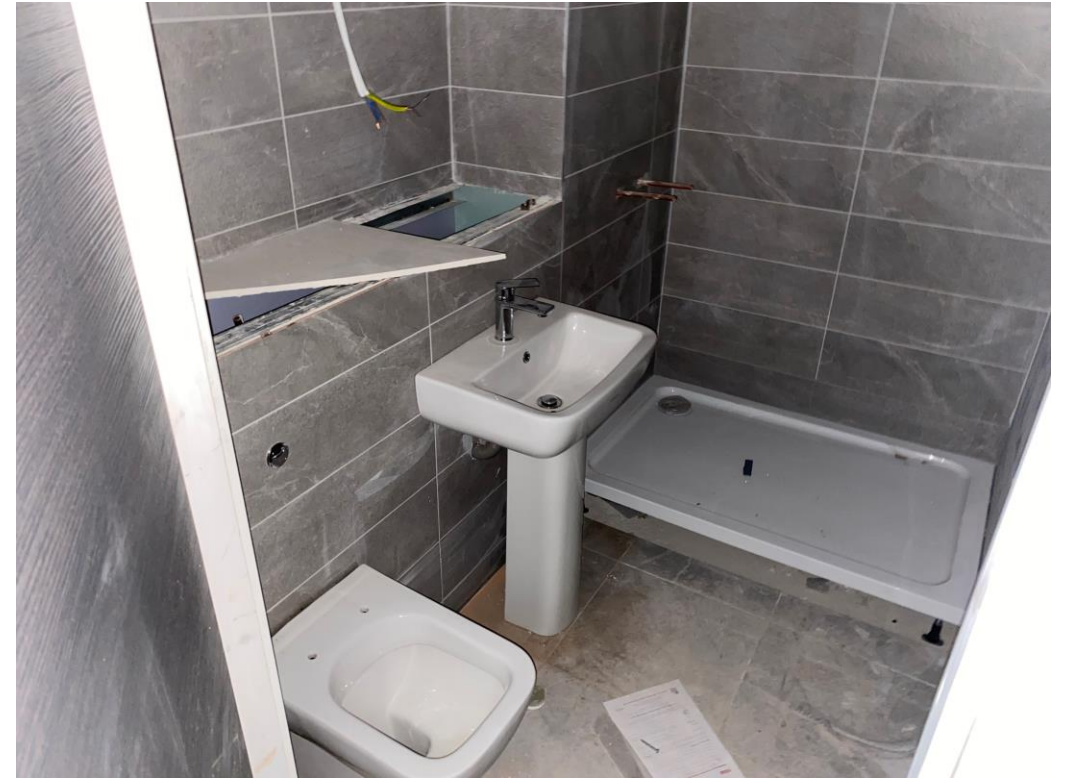
Residential Wing – Bathroom appliances on-going
