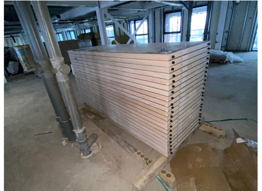
Material storage internal doors
