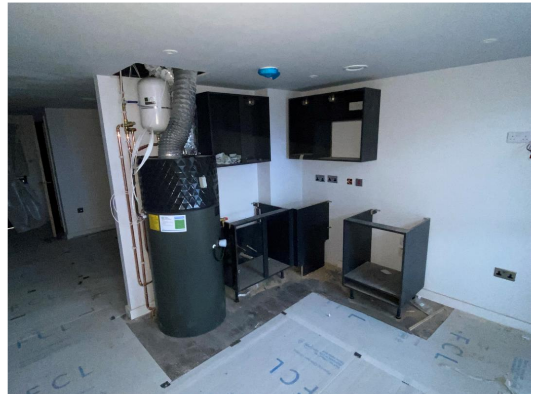
Residential Wing – KERS unit installation and Kitchen on-going
