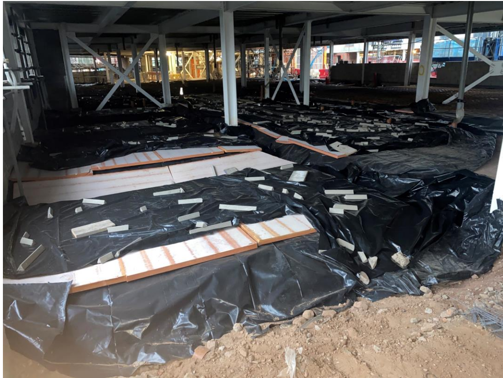
Residential Wing – Ground floor slab preparation ongoing
