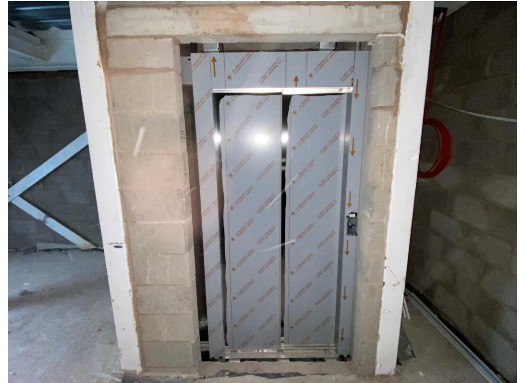
Student Wing – Lift installation
