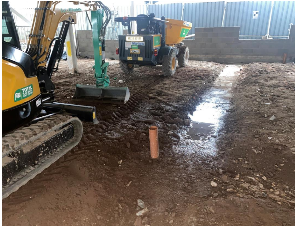
Residential Wing – Ground levelling and under ground drainage
