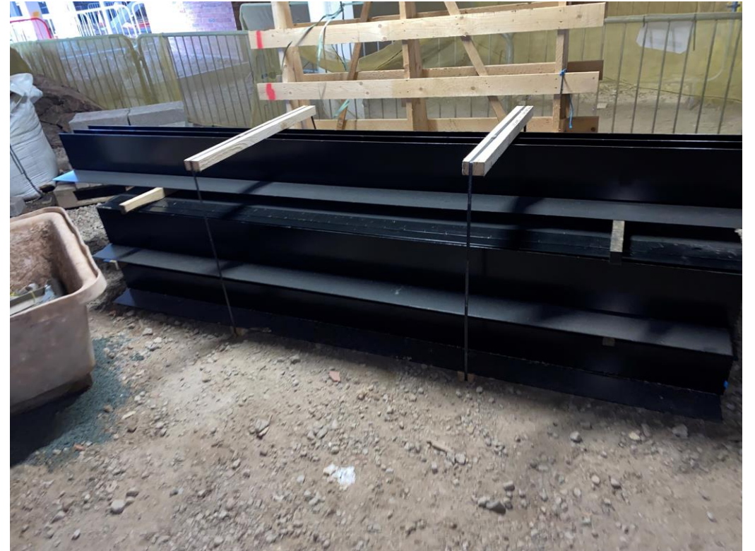
Material Storage – Steel lintels
