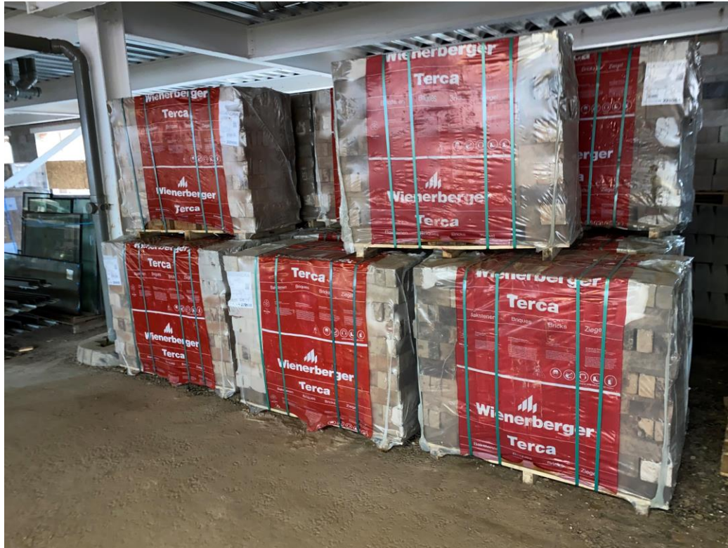
Material Storage – Wienerberger brick
