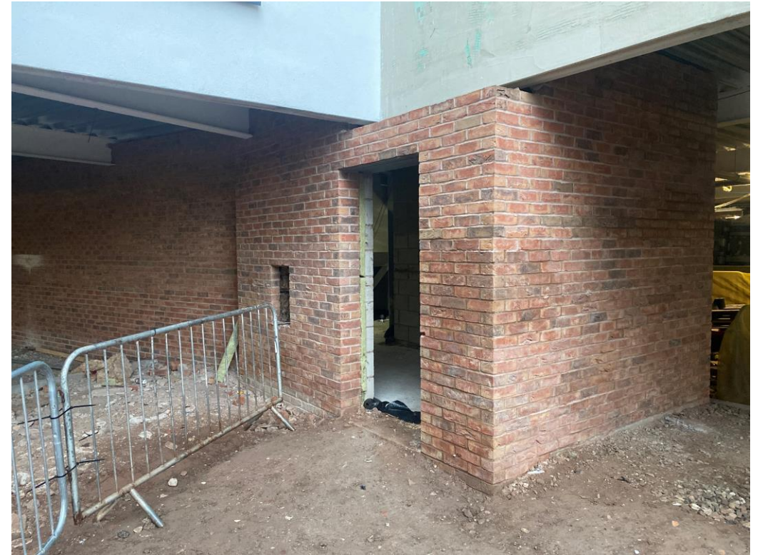
Student Wing – External brickwork
