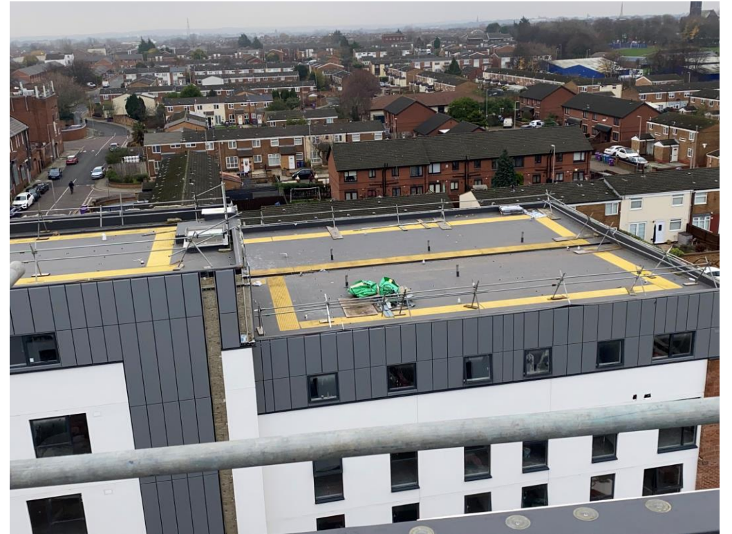
Student Wing – Roof works and cladding ongoing
