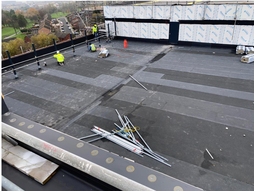
Commercial Block – Waterproofing to upstand columns
