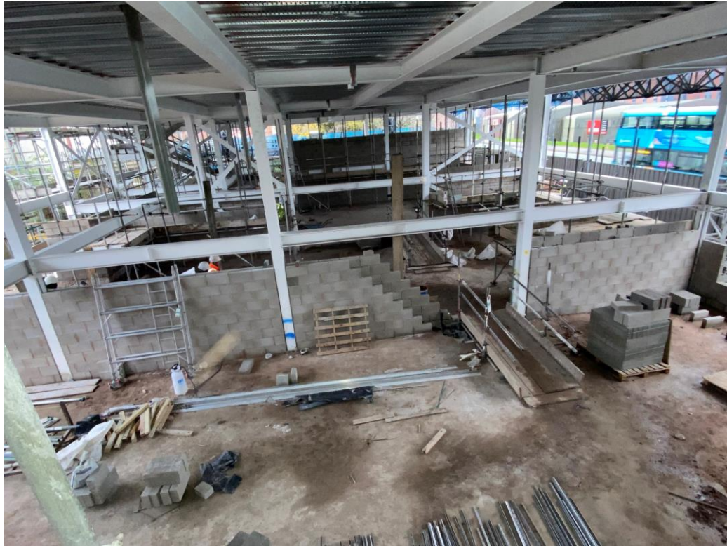
Commercial Units – General site activity
