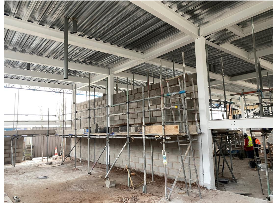
Residential Wing – Internal blockwork ongoing
