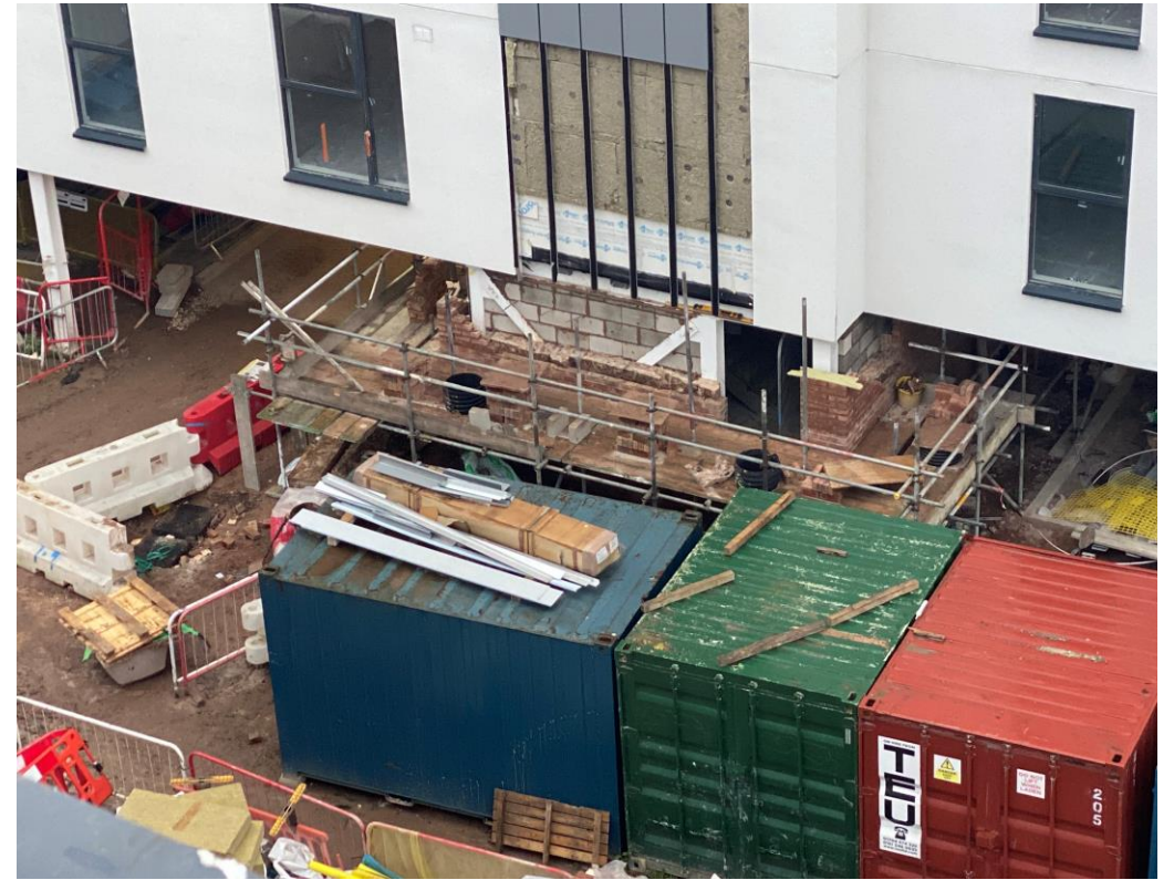
Student Wing – External brickwork and cladding ongoing
