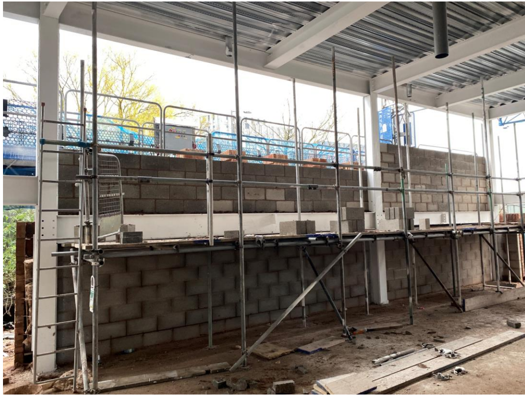
Residential Wing –Blockwork ongoing
