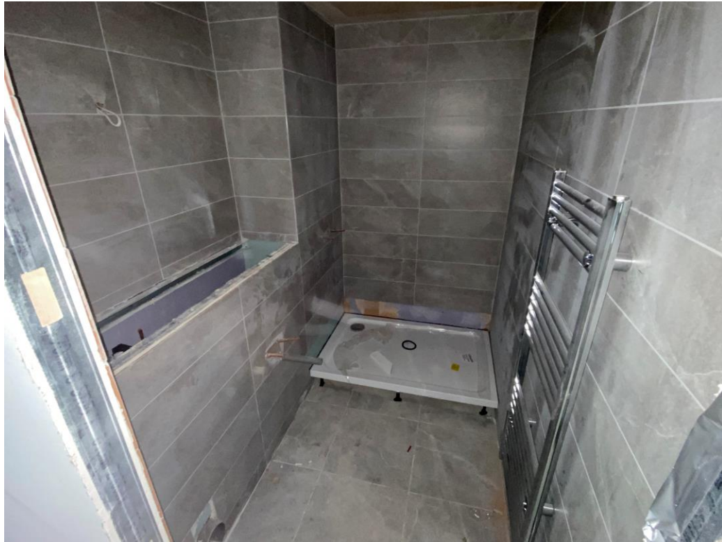
Residential Wing – Bathroom appliances on-going
