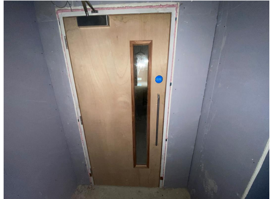
Student Wing – Internal door installation
