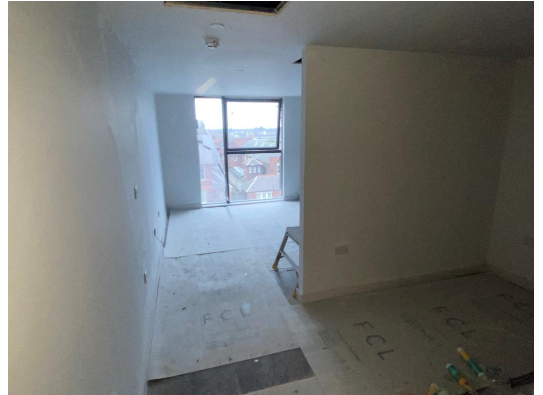
Student Wing – Internal finishes ongoing
