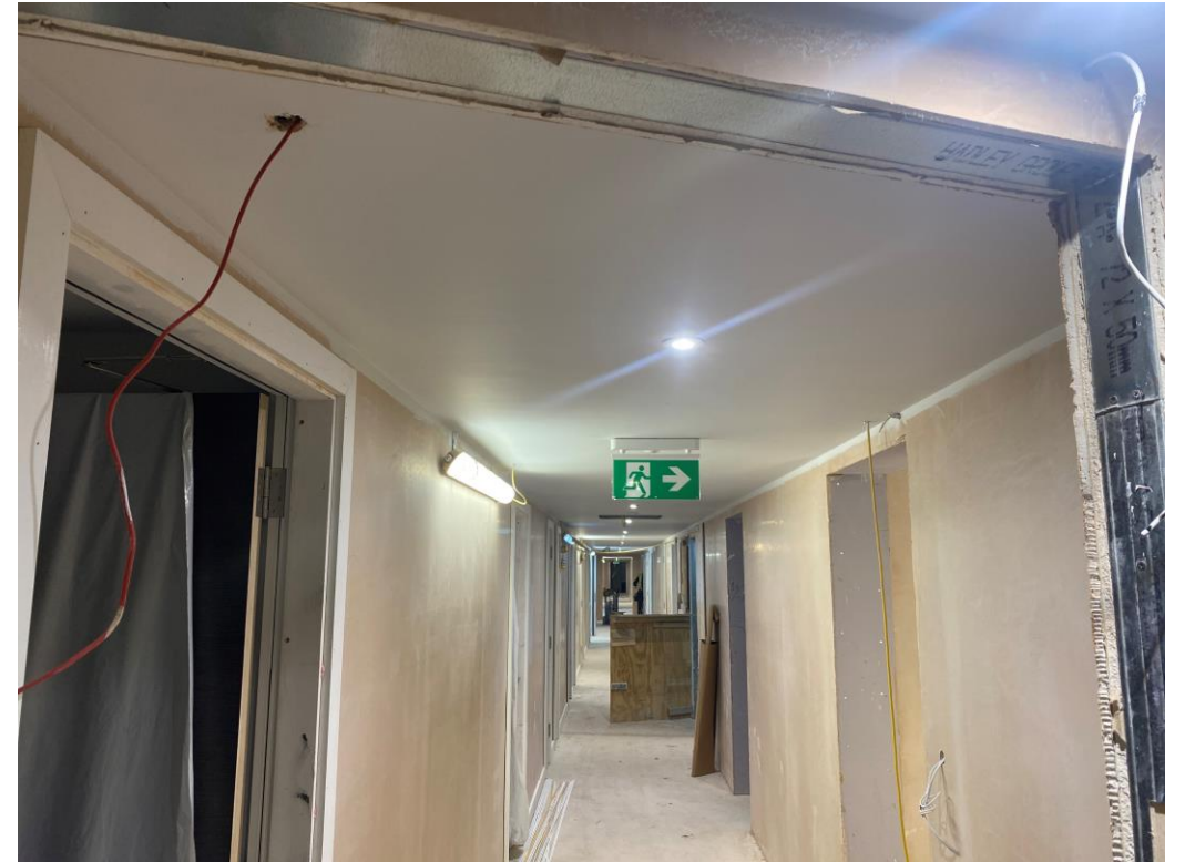
Student Wing – Internal finishes on-going
