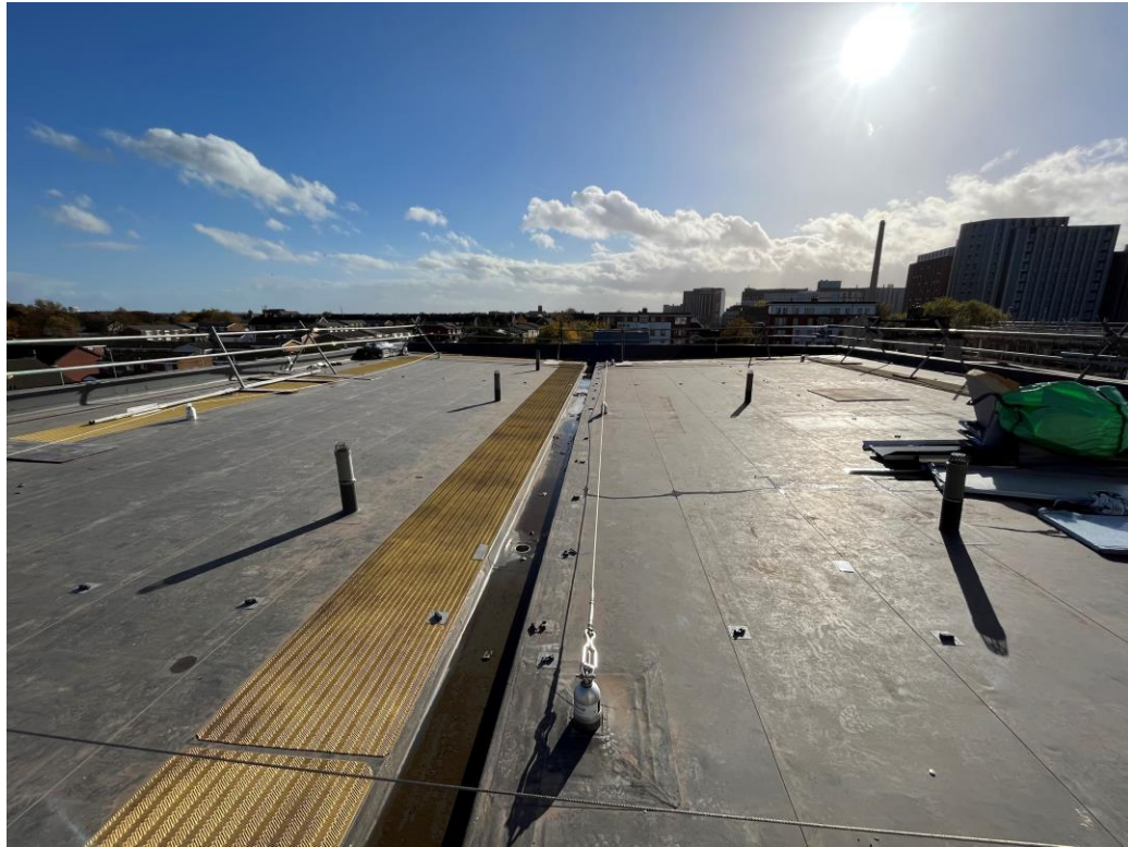
Student Wing – Mansafe system on-going
