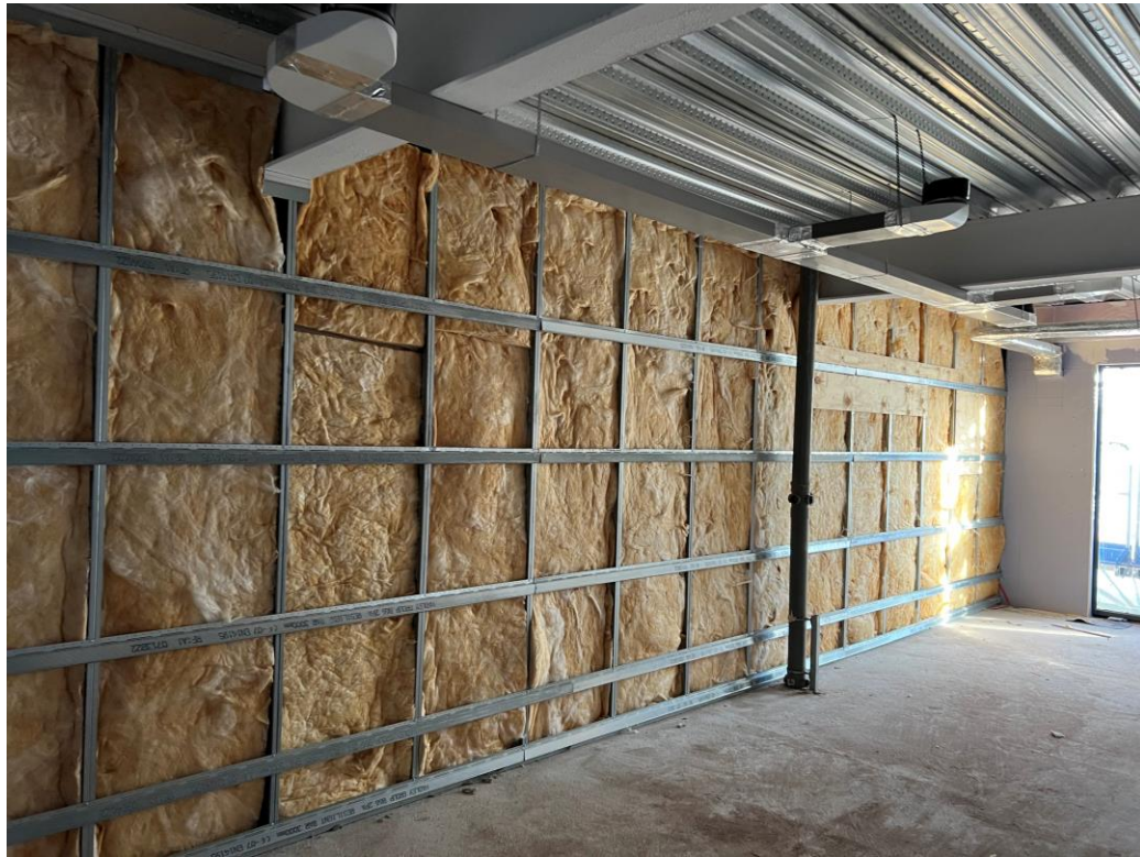
Residential Wing – Insulation and boarding of partition walls on-going
