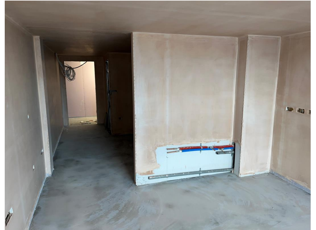
Student Wing – Plaster skim studio walls and ceilings
