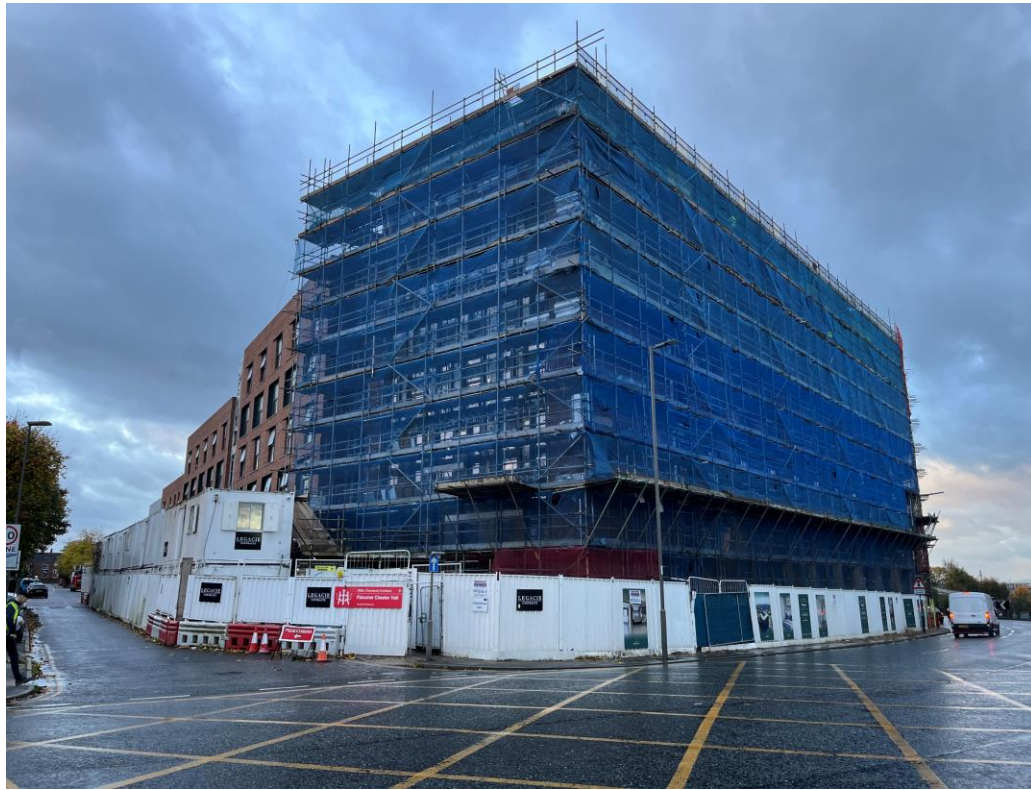
West Derby Road - Site view
