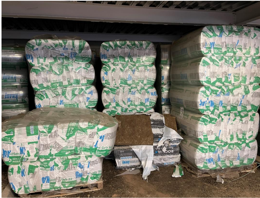
Material storage – Rockwool insulation
