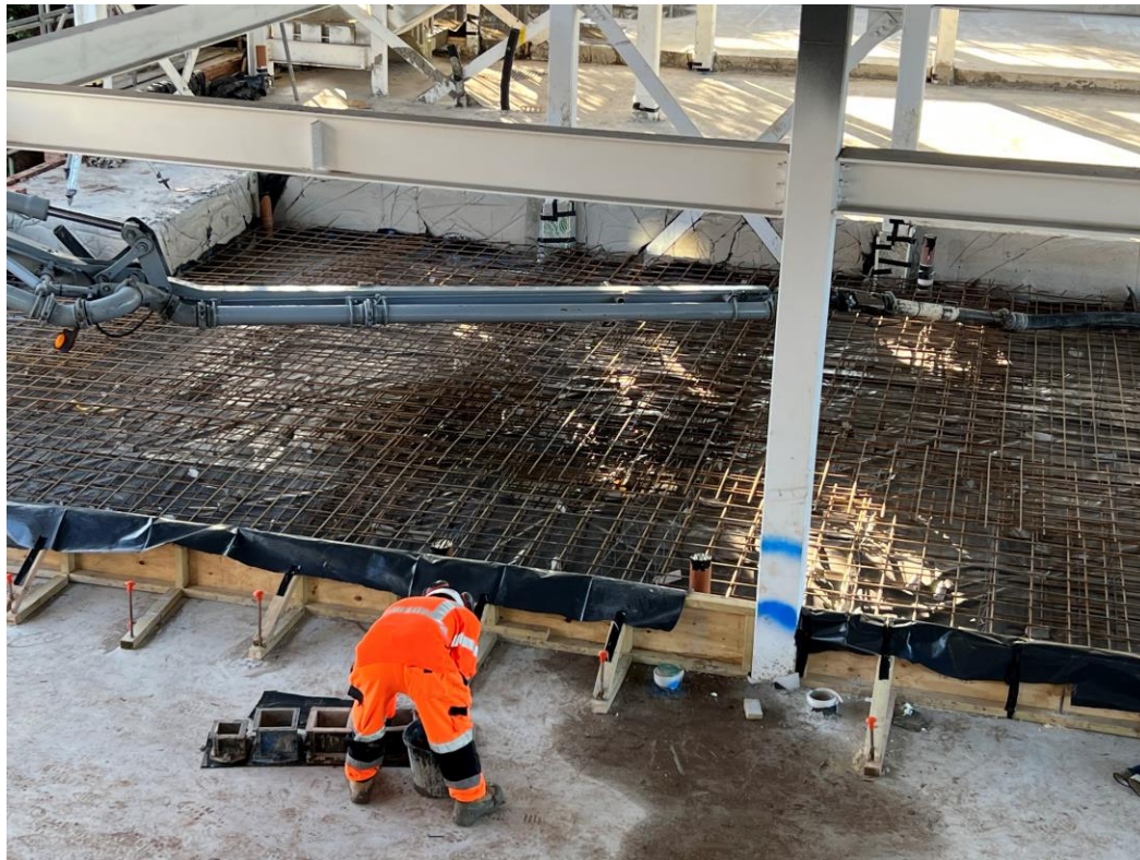
Commercial Block – Ground floor concrete slab preparations
