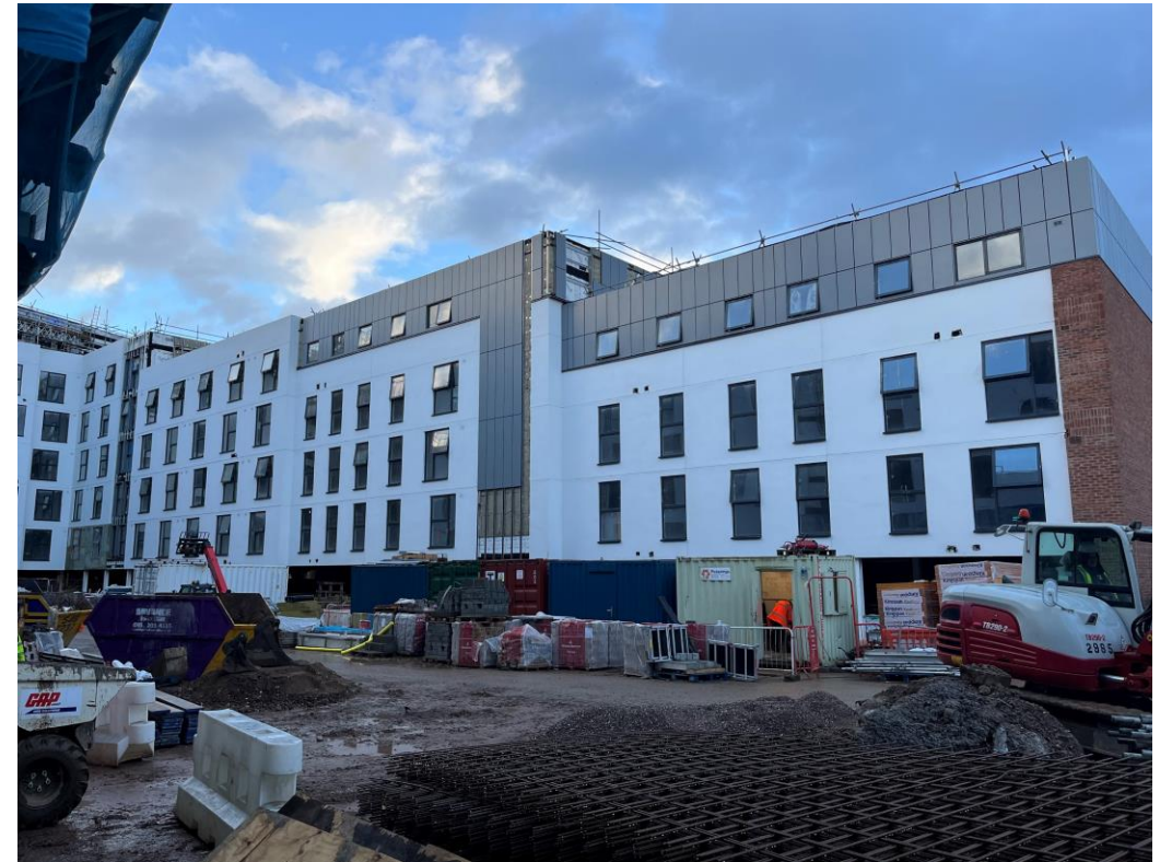
Student wing – Cladding installation ongoing
