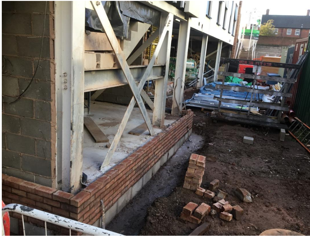
Student Wing – Brickwork to stair Core 5 on-going
