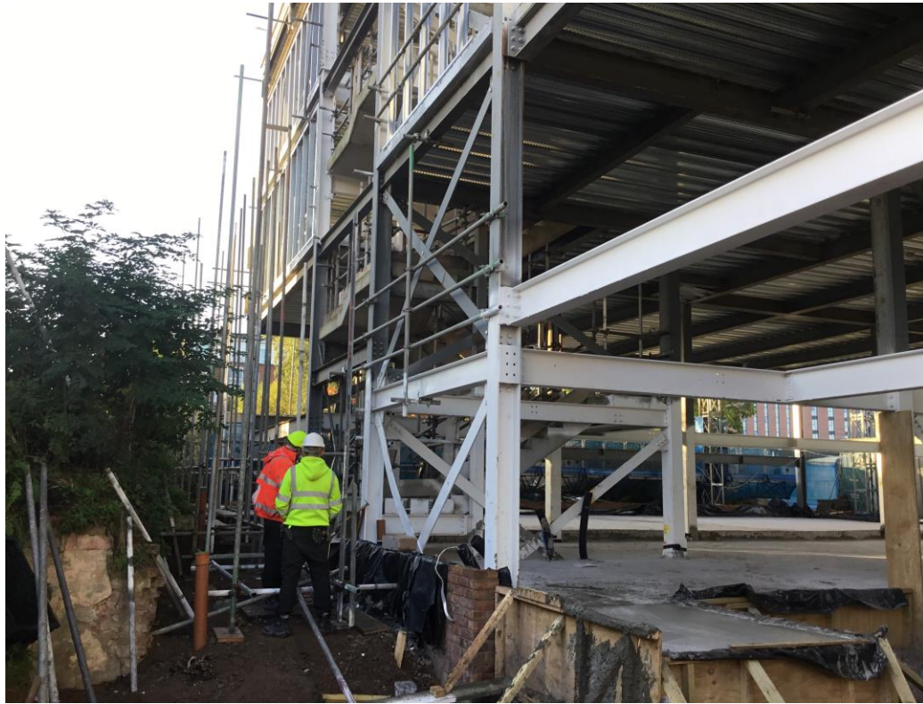
Commercial Block – Scaffolding erection commenced
