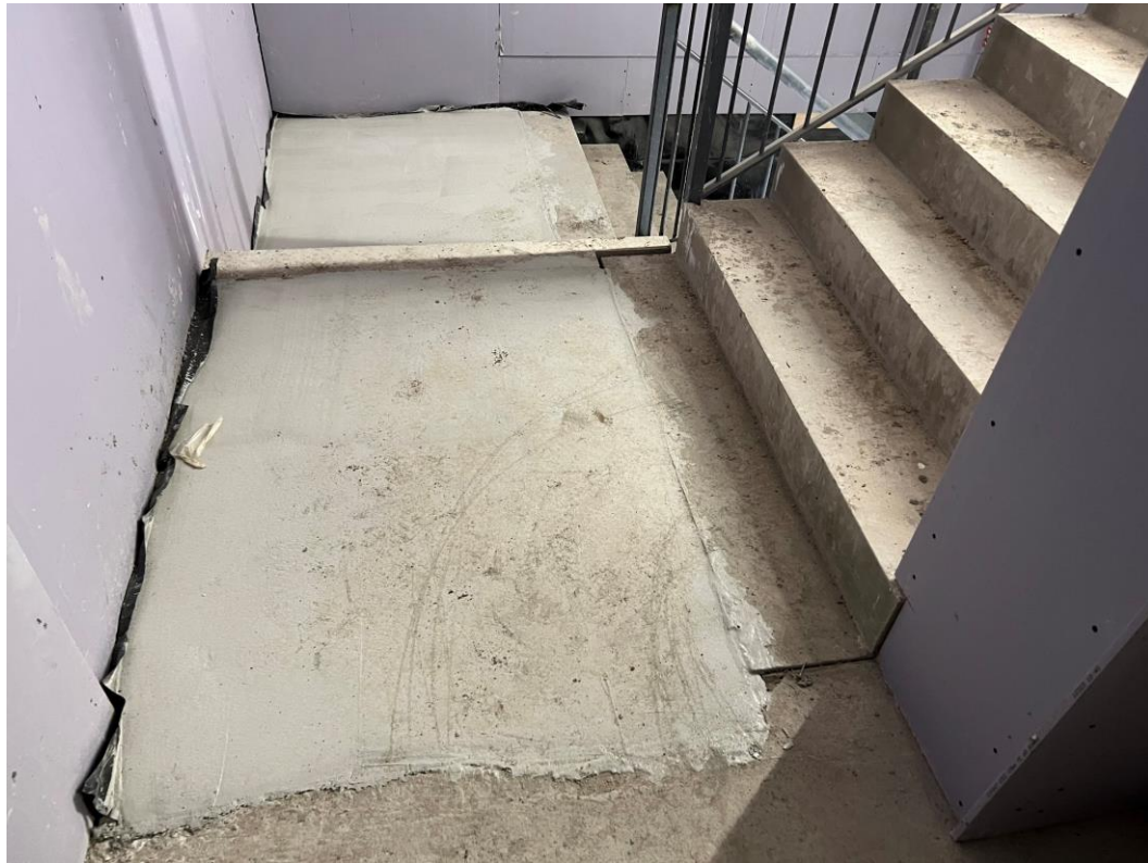
Stairwell floor screed installed
