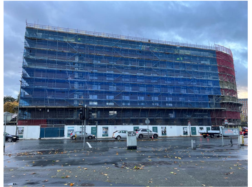
West Derby Road - Site view
