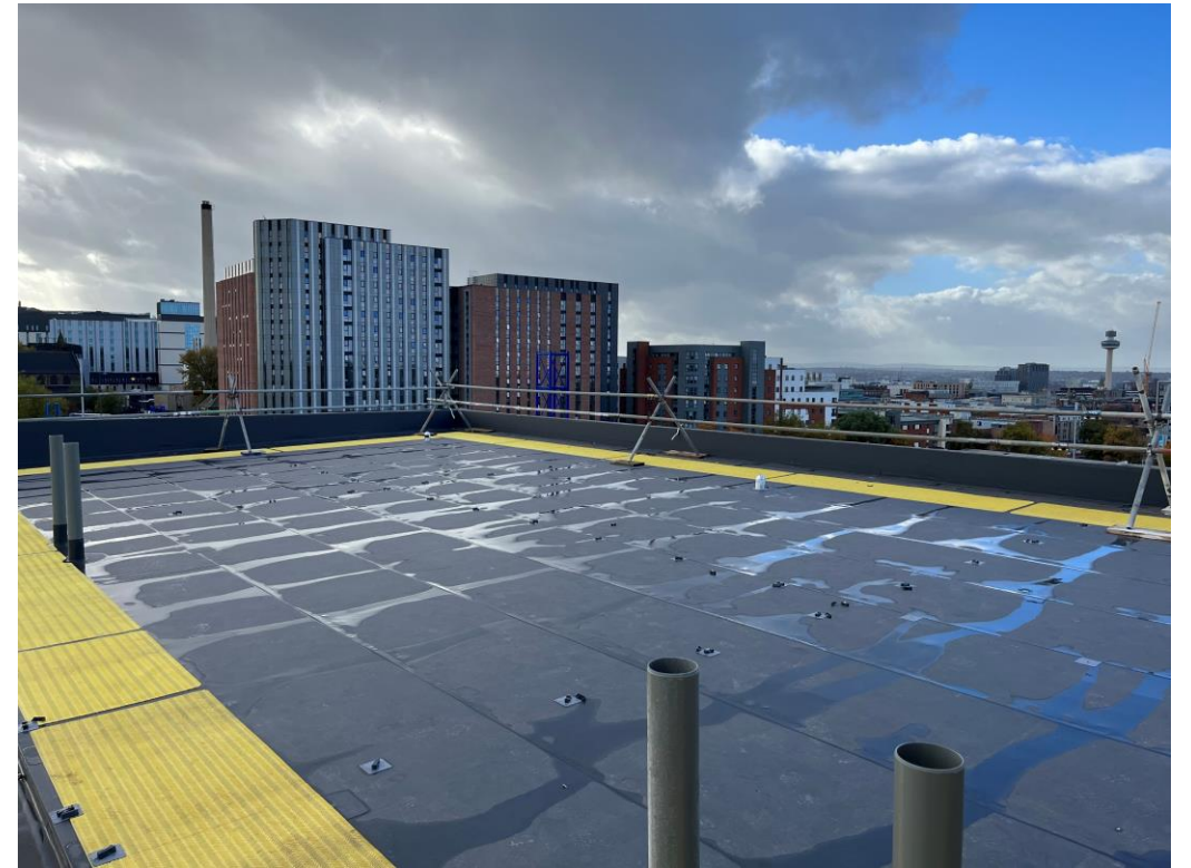
Commercial Block – Temporary edge protection
