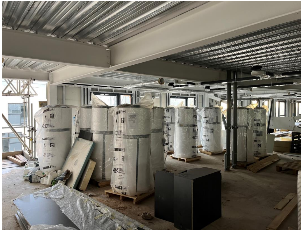
Material storage – KERS units
