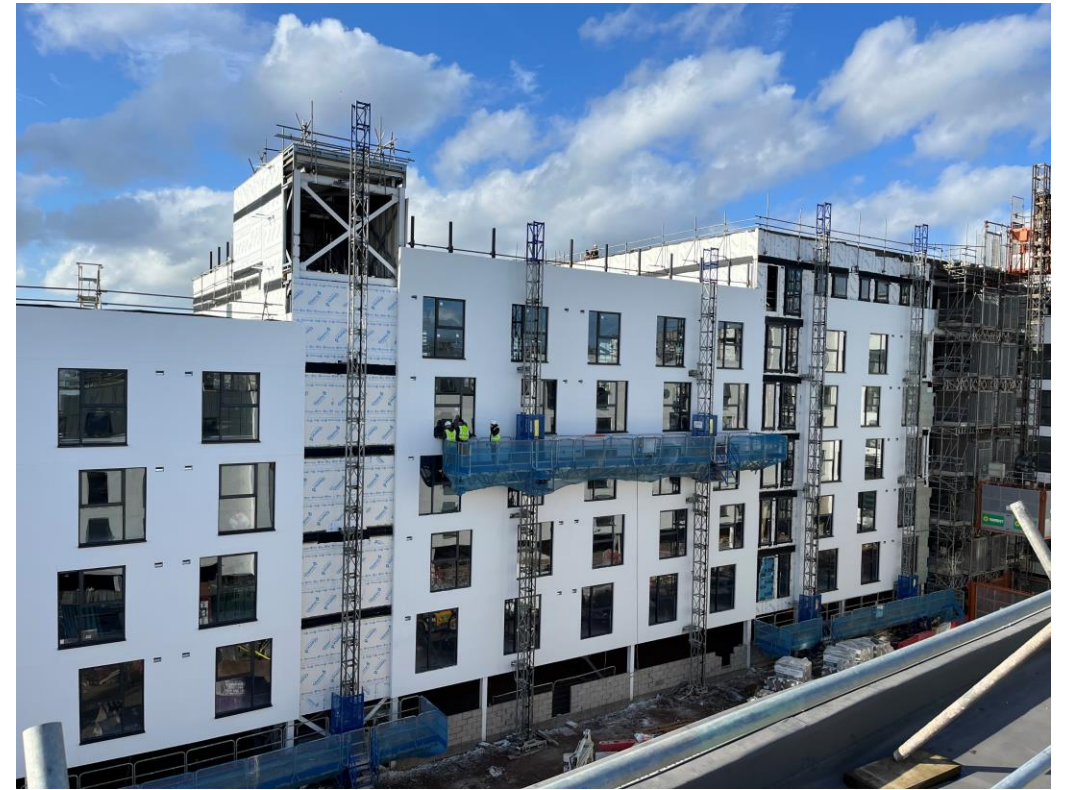
Residential Wing – Render coat decorated to inner courtyard elevation
