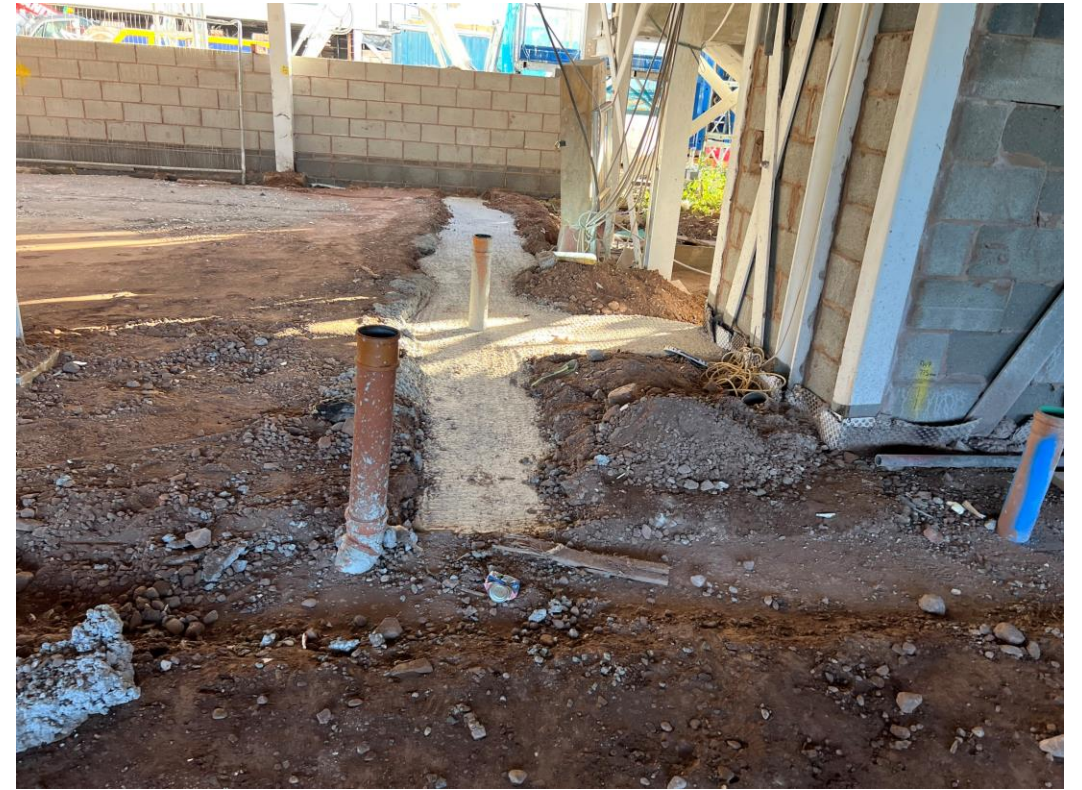
Communal area – Ground floor slab preparation
