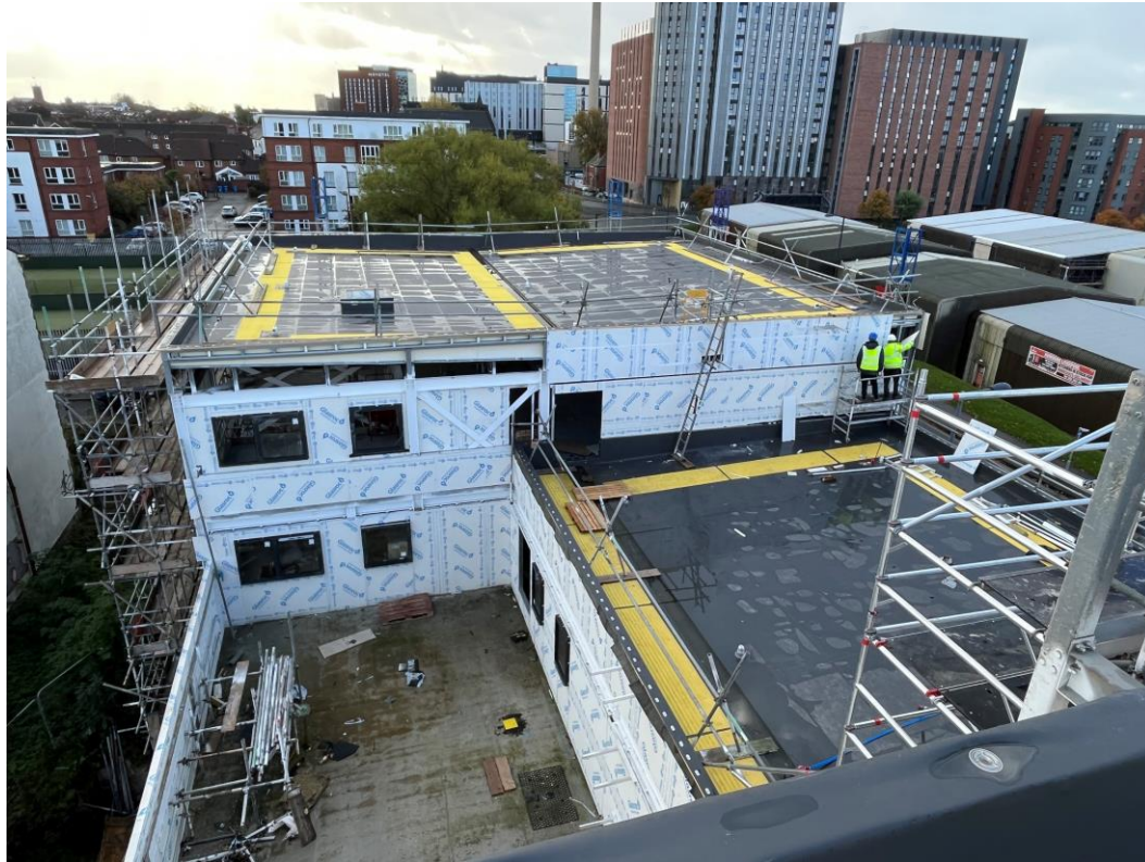
Commercial Block – Weatherboarding on-going
