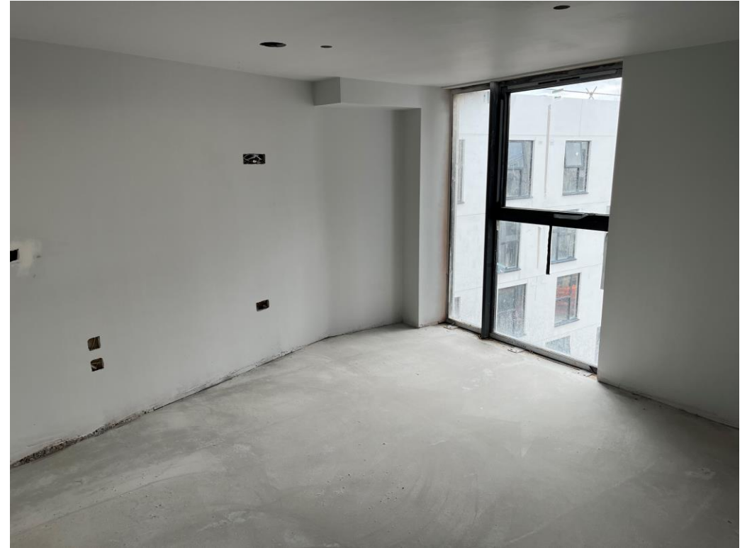
Residential Wing – Internal finishes on-going
