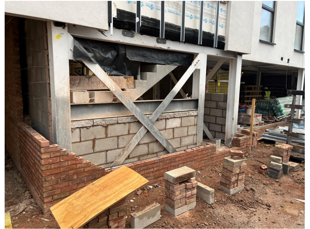
Student Wing – Brickwork and blockwork to stair Core 5 Progress
