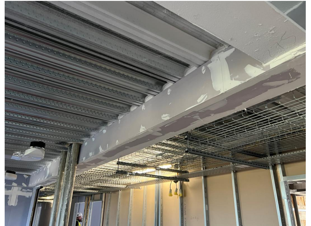
Residential Wing – Fire stopping works and cable trays on-going
