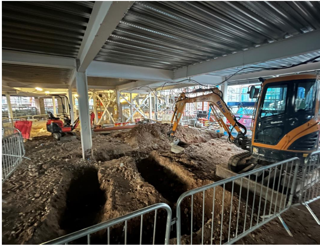
Residential Block – Under ground drainage works on-going
