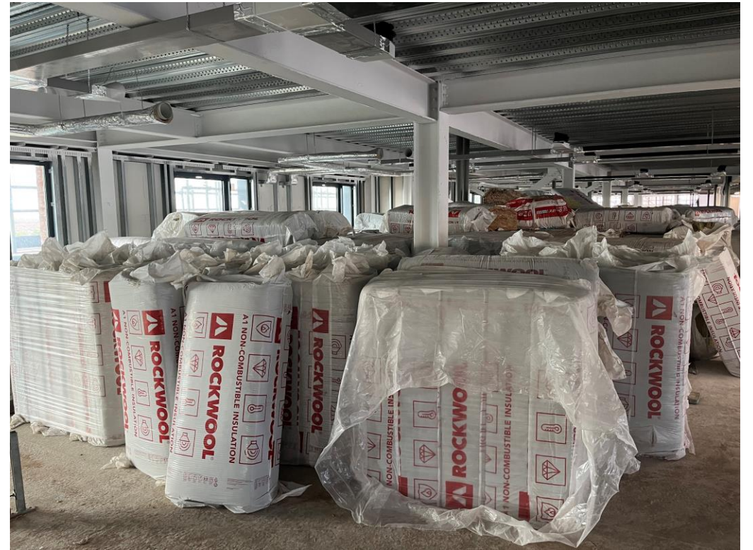
Material storage – Rockwool insulation
