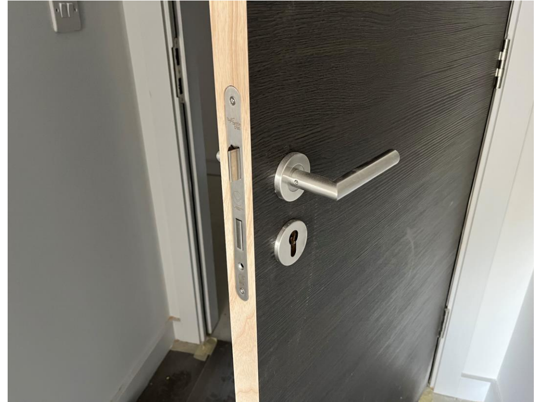
Student Wing – Ironmongery installation on-going
