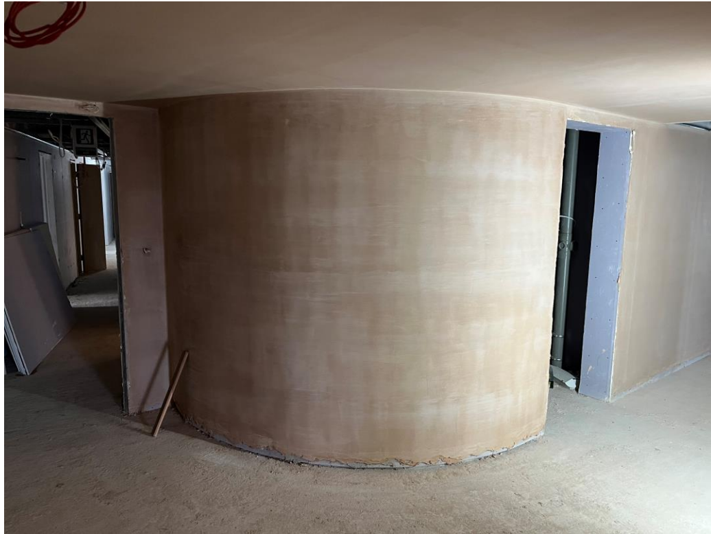
Residential Wing – Plaster work on-going
