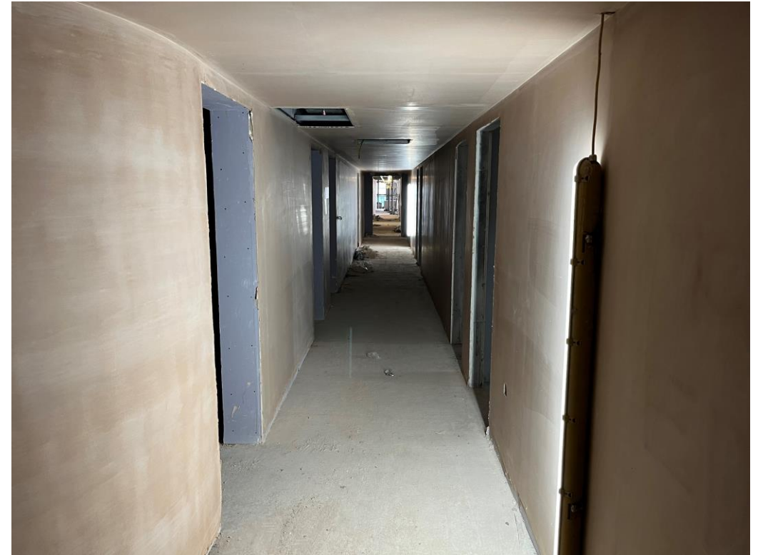
Residential Wing – Plaster work on-going
