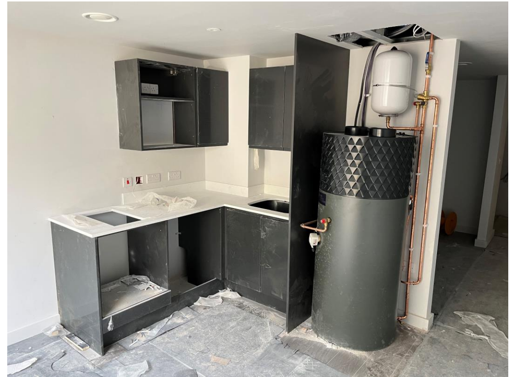
Student Wing – Kitchen on-going and KERS unit installation
