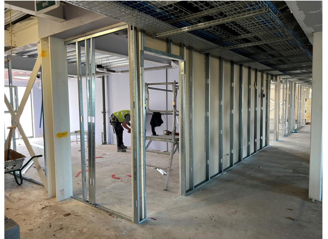
Residential Wing – Erection and boarding of partition walls
