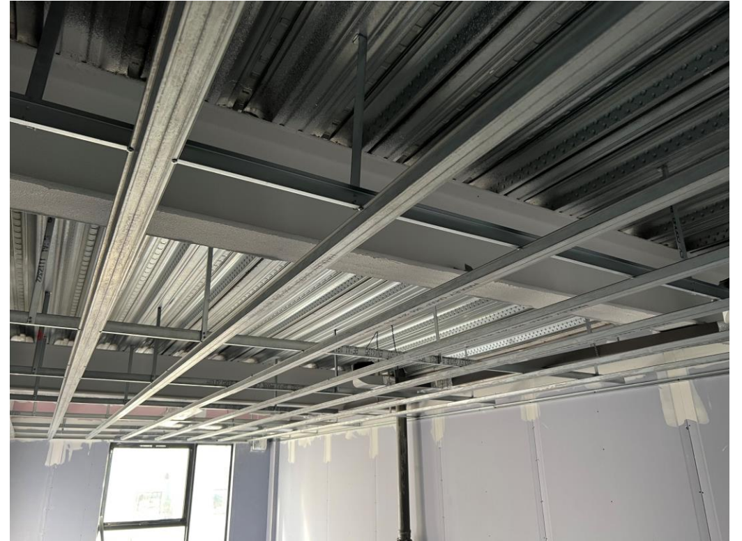
Residential Wing– Metal ceiling grid on-going
