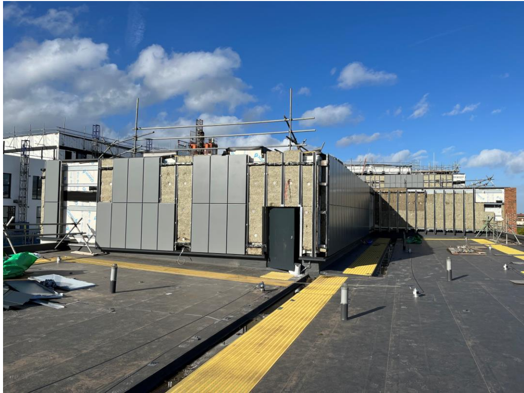
Student Wing – External insulation and cladding on-going
