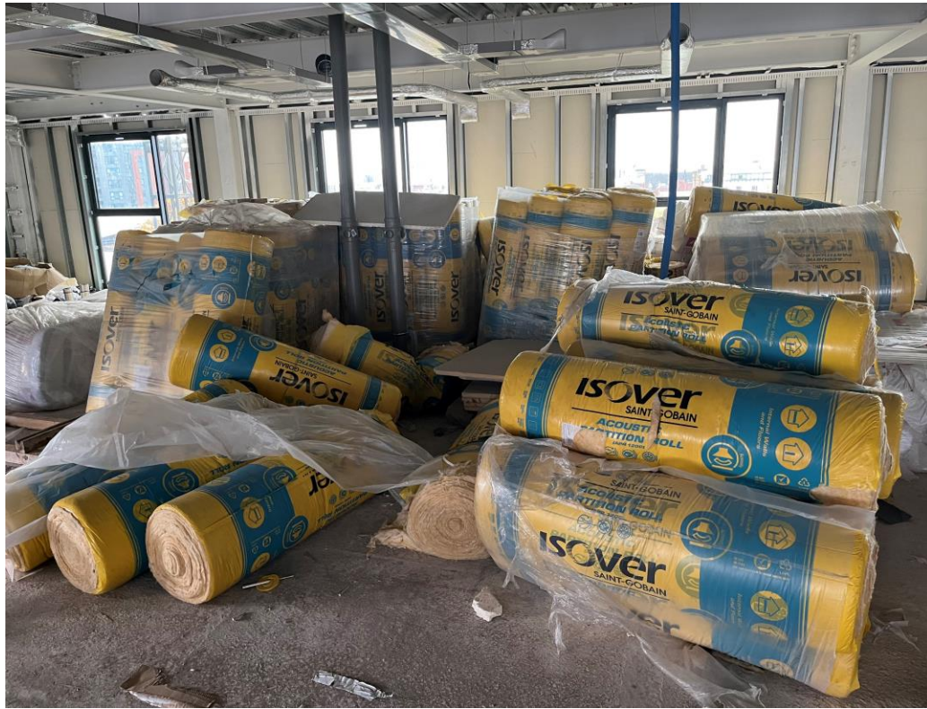
Material storage - Acoustic partition roll
