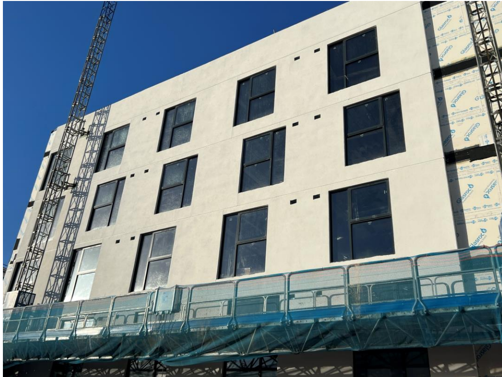
Residential Wing – Render coat applied to inner courtyard elevation
