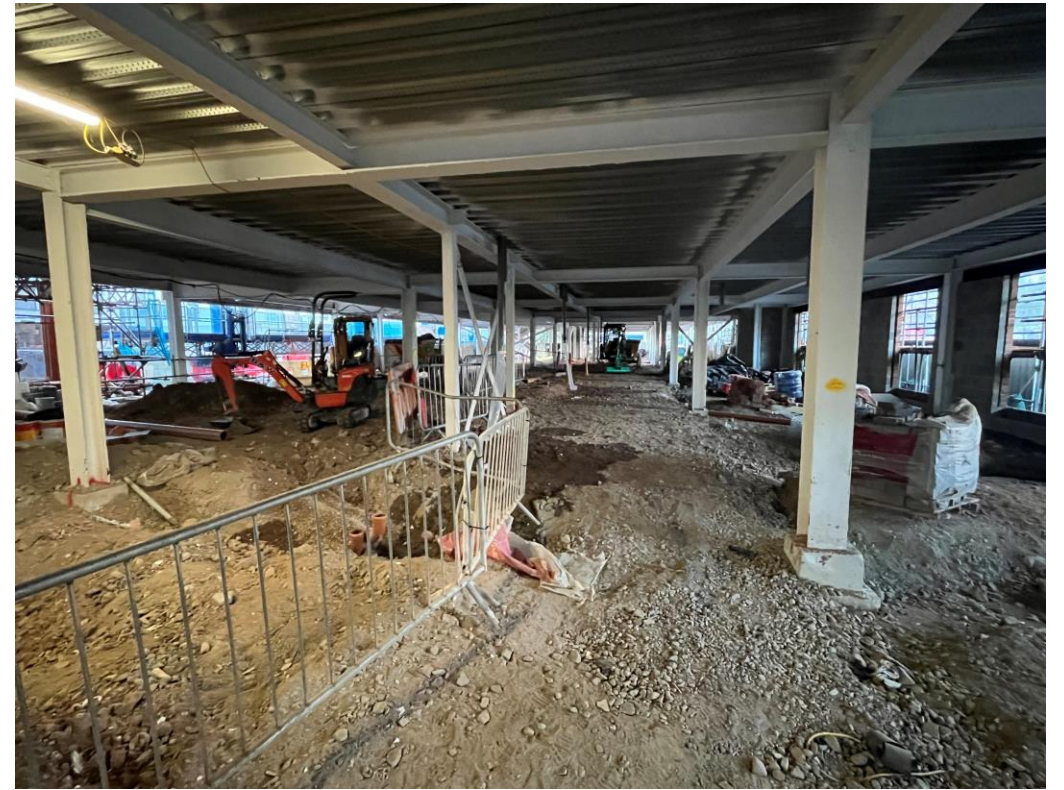
Residential Block – Under ground drainage works and ground levelling
