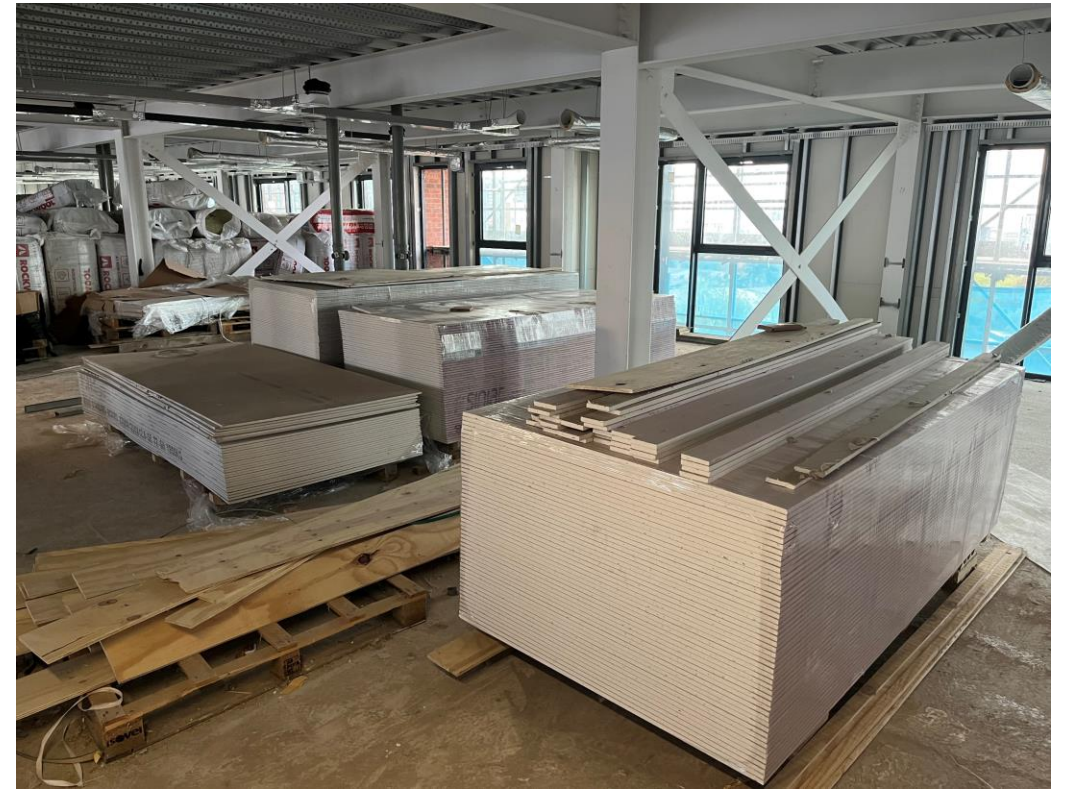
Material storage – Skirting boards
