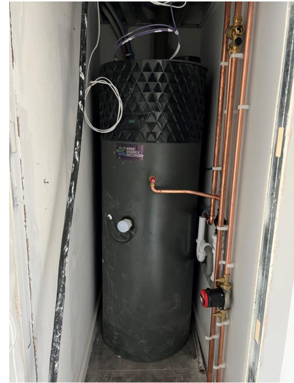
Student Wing – KERS unit installation
