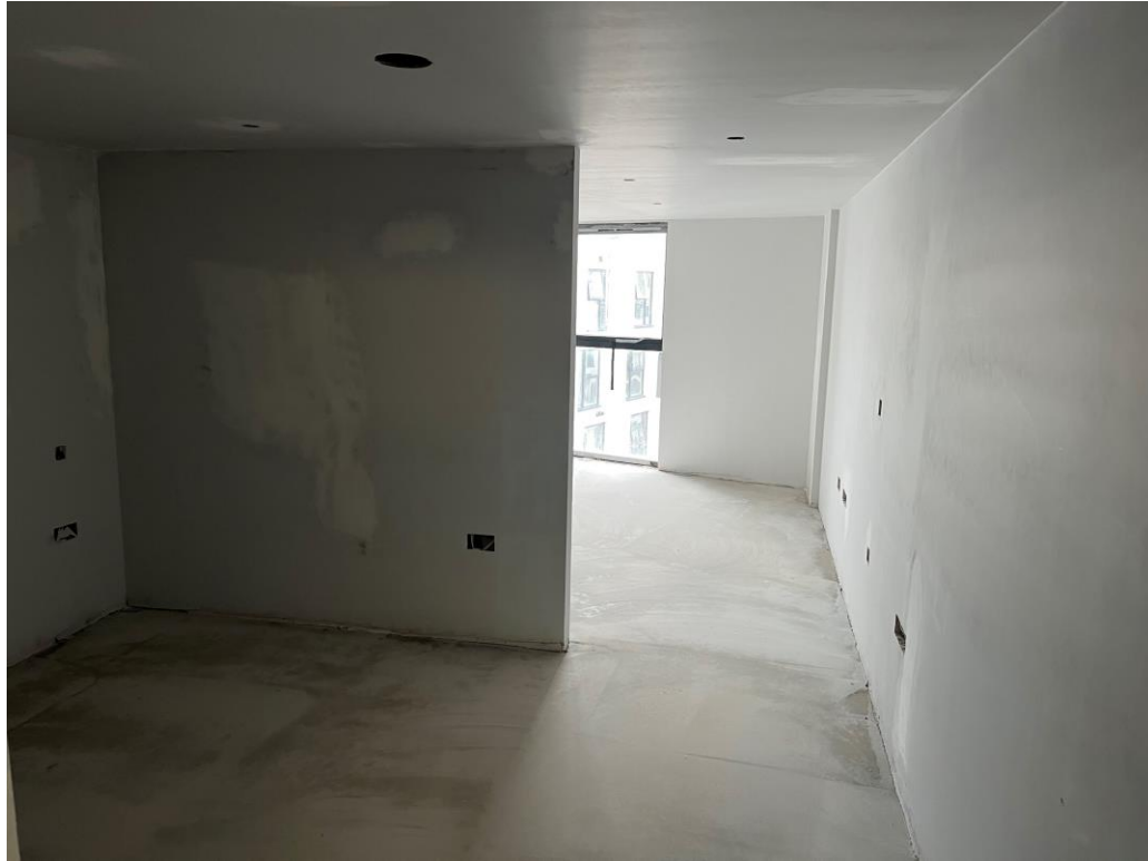
Residential Wing – Internal finishes on-going
