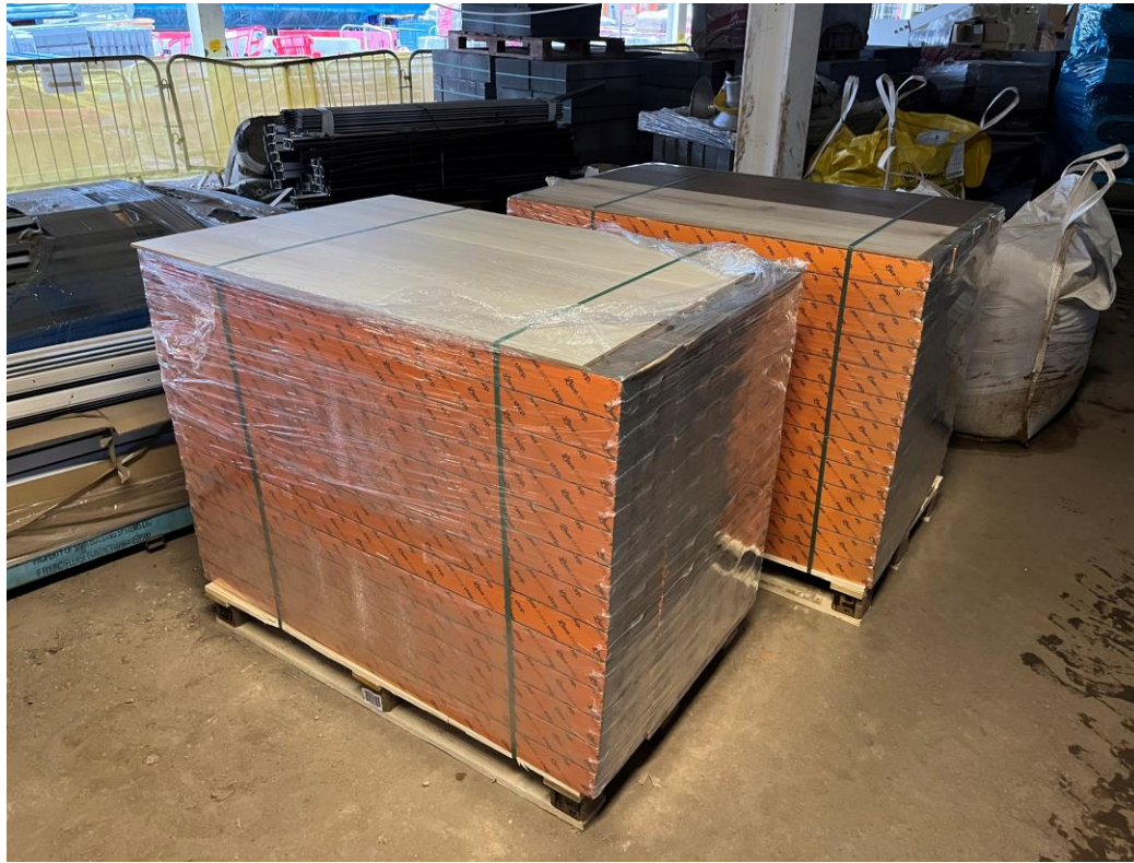
Material storage – Laminate flooring
