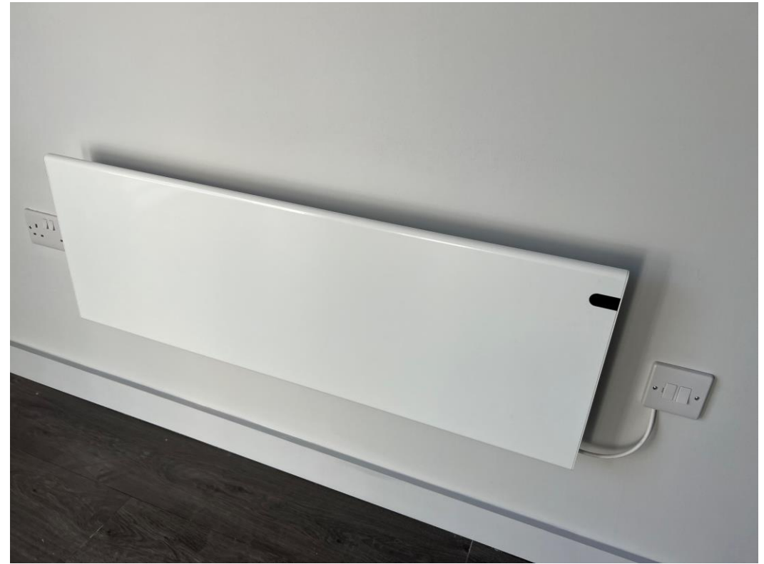
Student Wing – Panel wall heater installed
