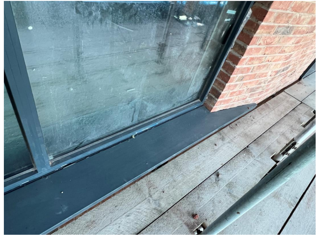
Residential wing – External elevation brickwork on-going
