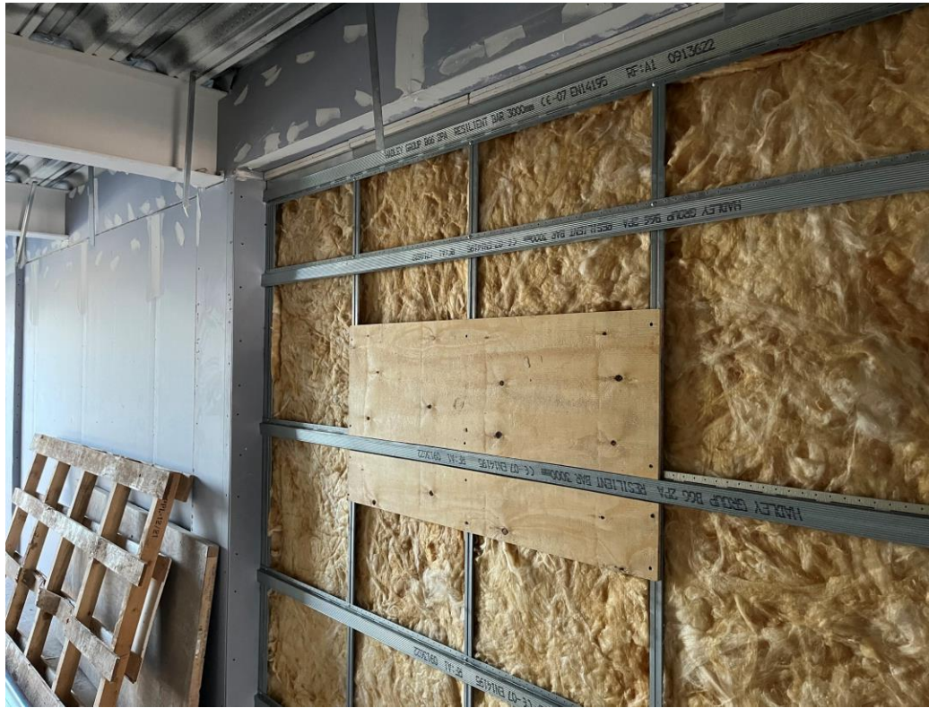
Residential Wing – Pattress, insulation and boarding of walls
