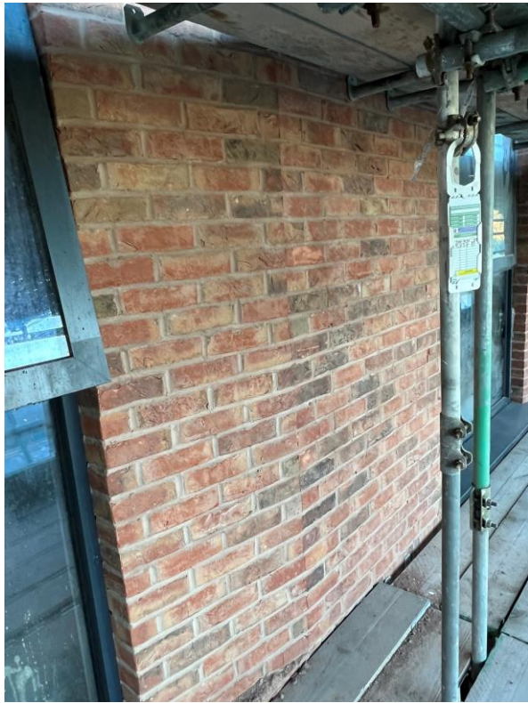
Residential wing – External elevation brickwork on-going
