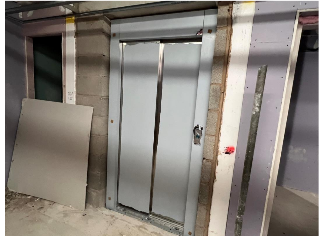
Student Wing – Lift installation
