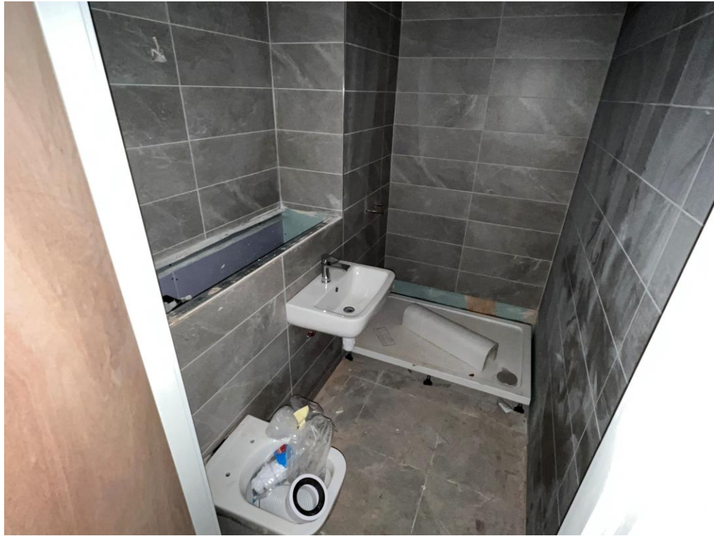
Student Wing – Bathroom appliances on-going
