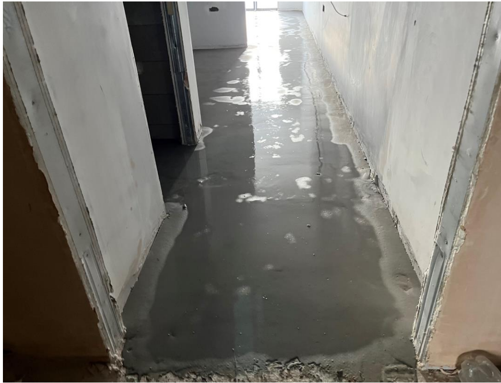
Residential Wing – Latex screed on-going
