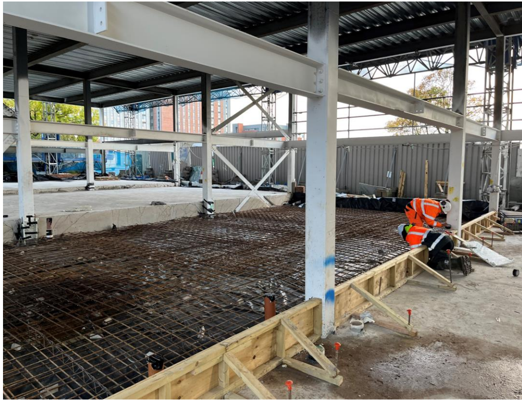
Commercial Block – Ground floor slab rebar installation
