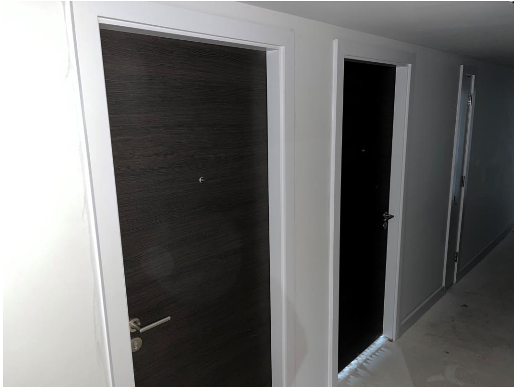
Student Wing – Internal doors and Ironmongery on-going
