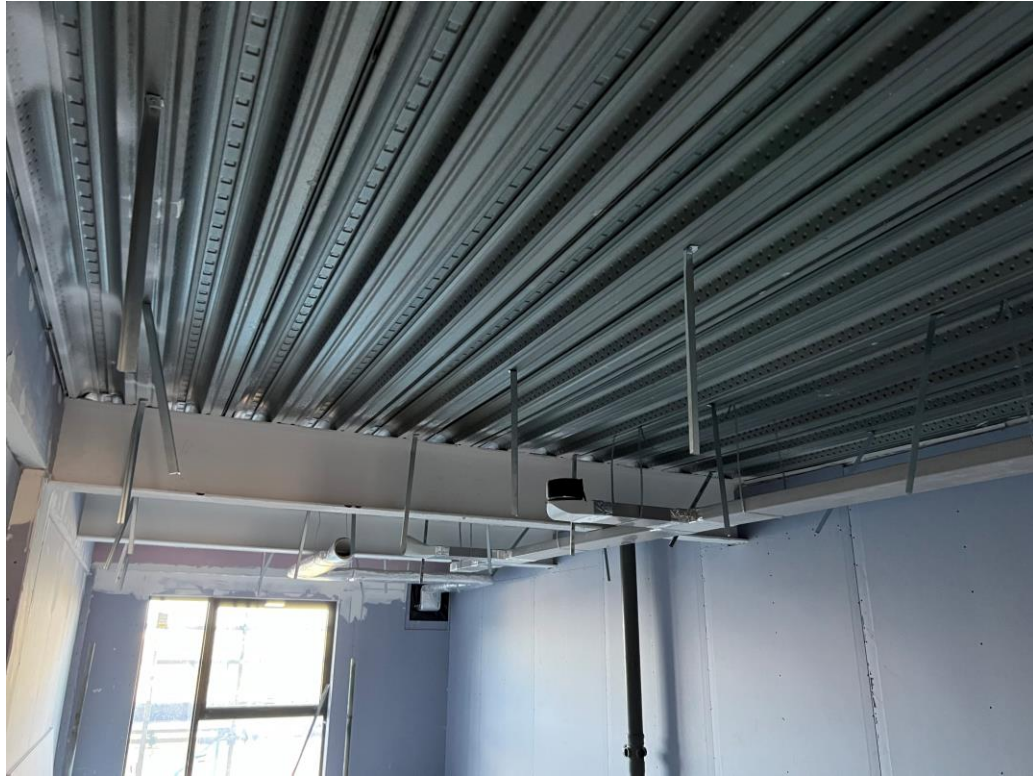
Residential Wing– Metal ceiling grid on-going
