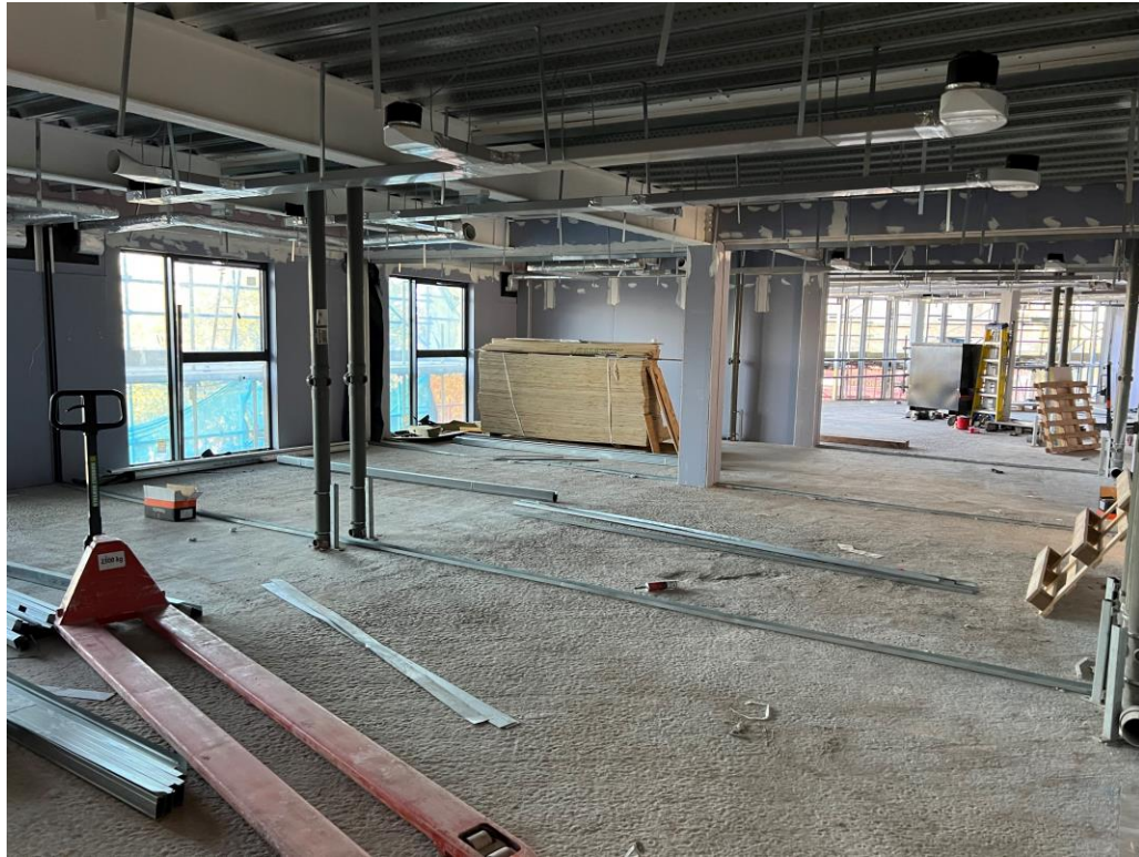
Residential Wing – Setting out partitions
