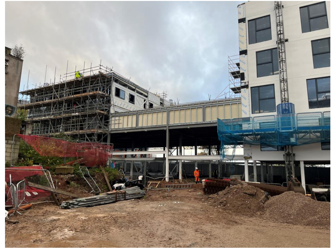
Commercial Block – Scaffolding erection on-going
