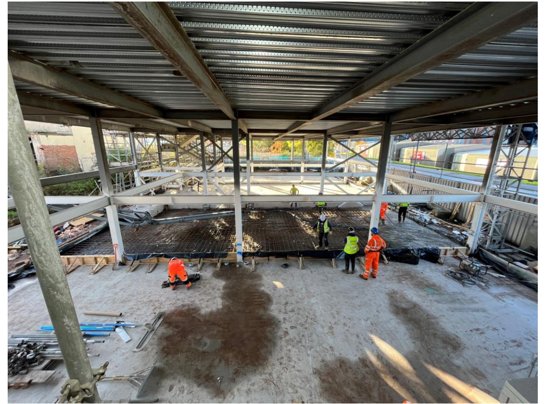
Commercial Block – Rebar installation and concrete slab pour
