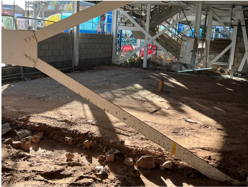
Communal area – Ground floor slab preparation
