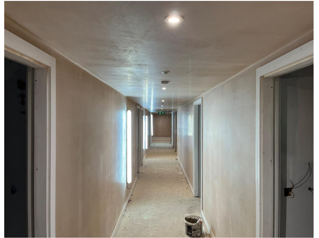
Residential Wing – Plaster skim walls and ceilings on-going
