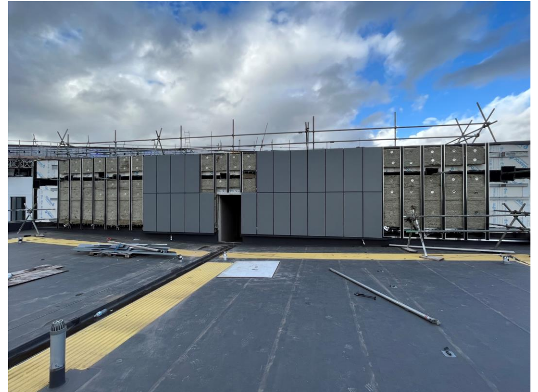
Student Wing – External insulation and cladding on-going
