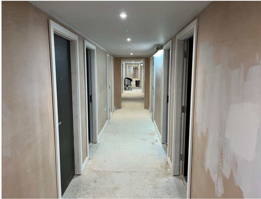
Student Wing – Internal finishes on-going
