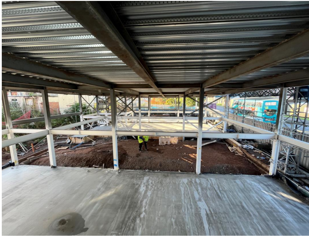
Commercial Block – Ground floor concrete slab preparations
