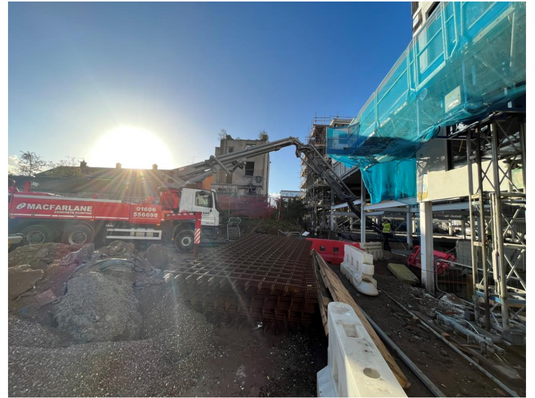
Commercial Block – Ground floor concrete slab pour
