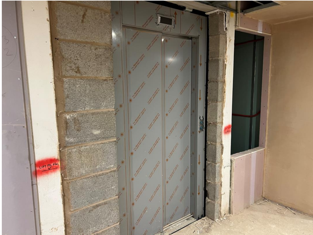
Student Wing – Lift installation
