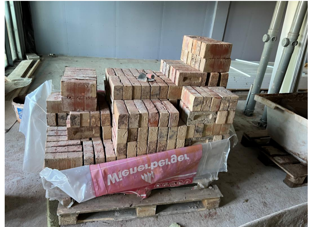
Material storage – Red brick
