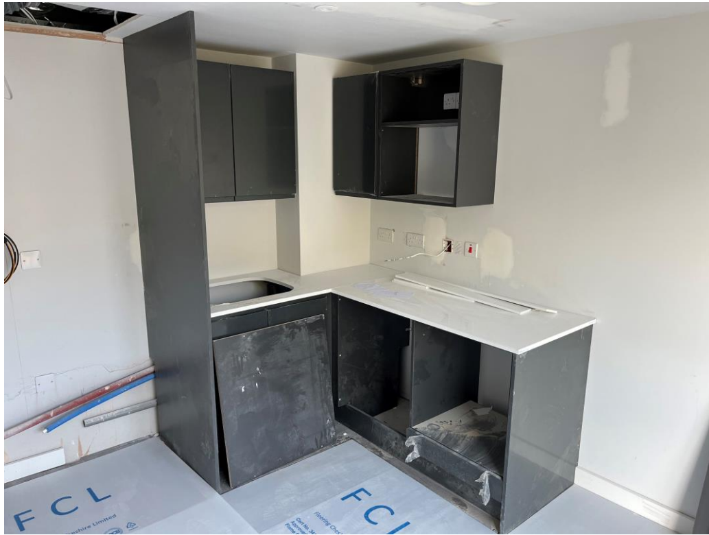
Student Wing – Kitchen on-going
