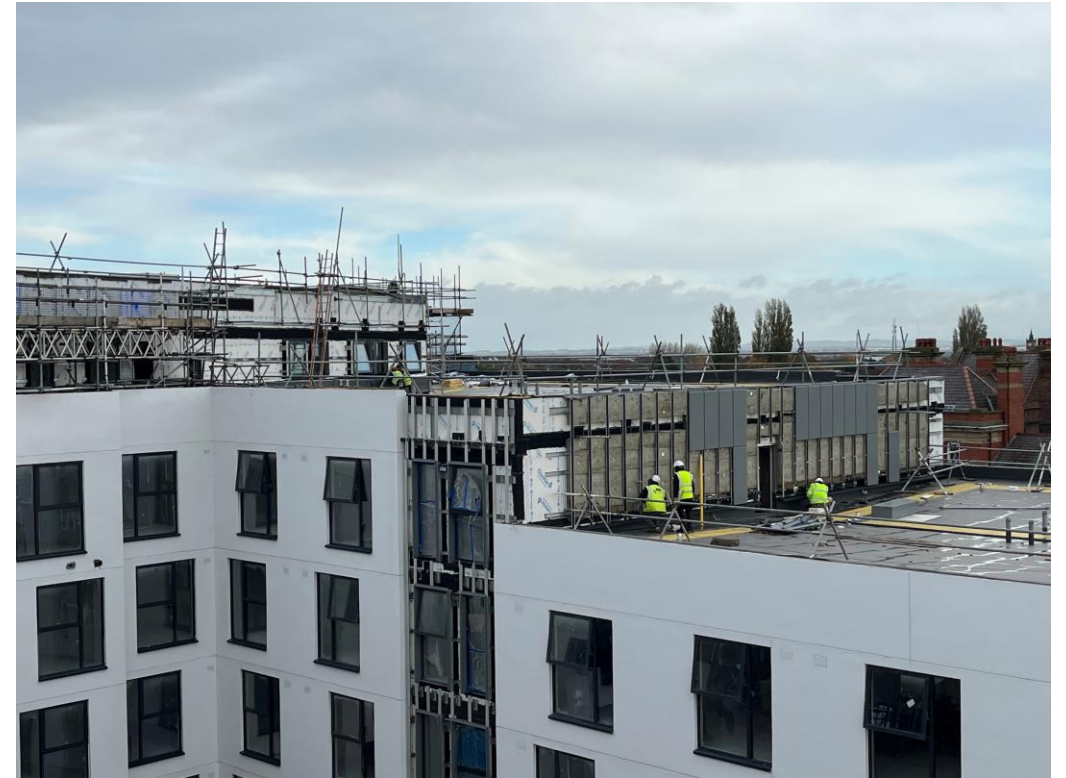
Student Wing – External insulation and cladding on-going
