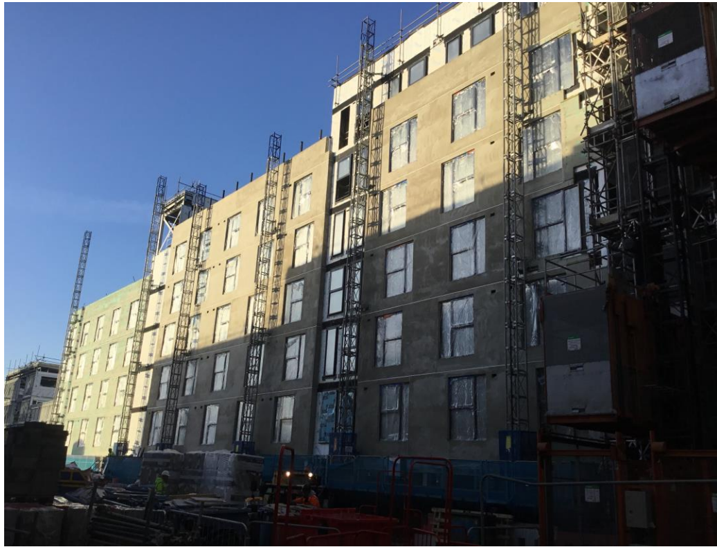
Residential Wing – Render coat applied to inner courtyard elevation
