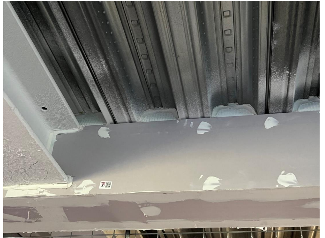
Fire stopping works
