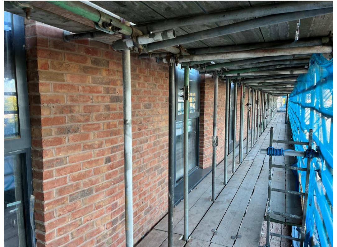
Residential wing – External elevation brickwork on-going
