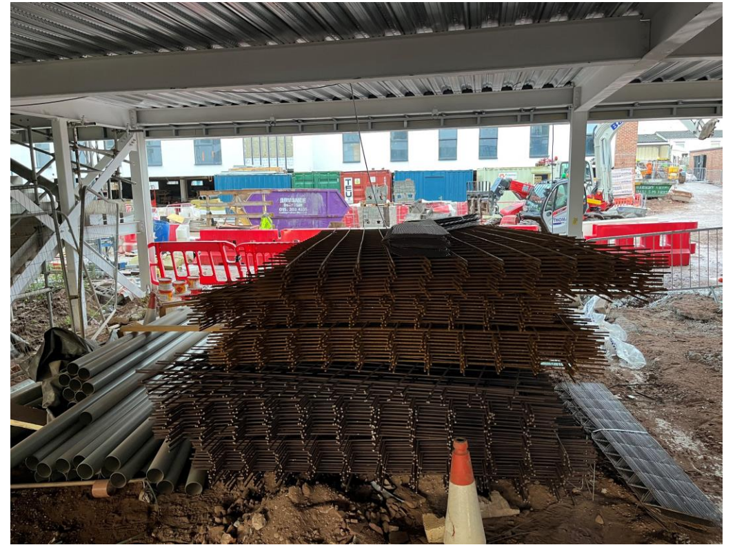
Material storage – Steel reinforcement
