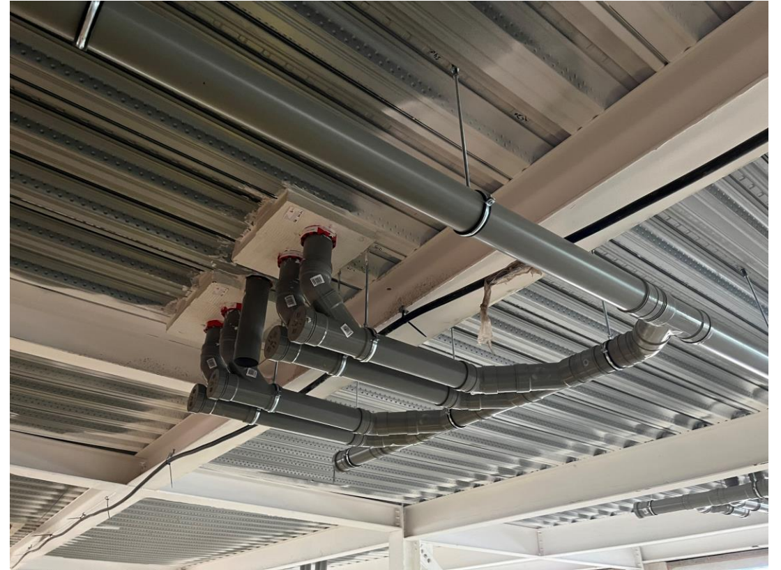
Residential Wing – Fire stopping works
