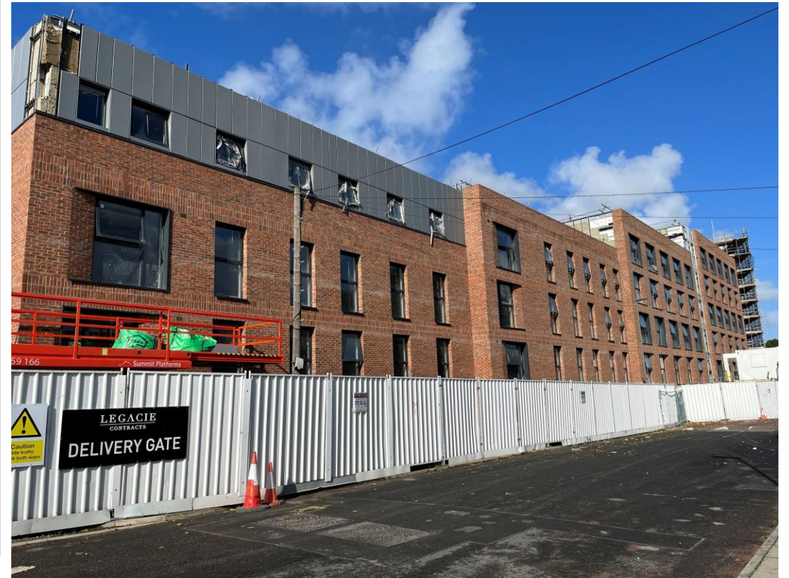
Walker Street - Site view
