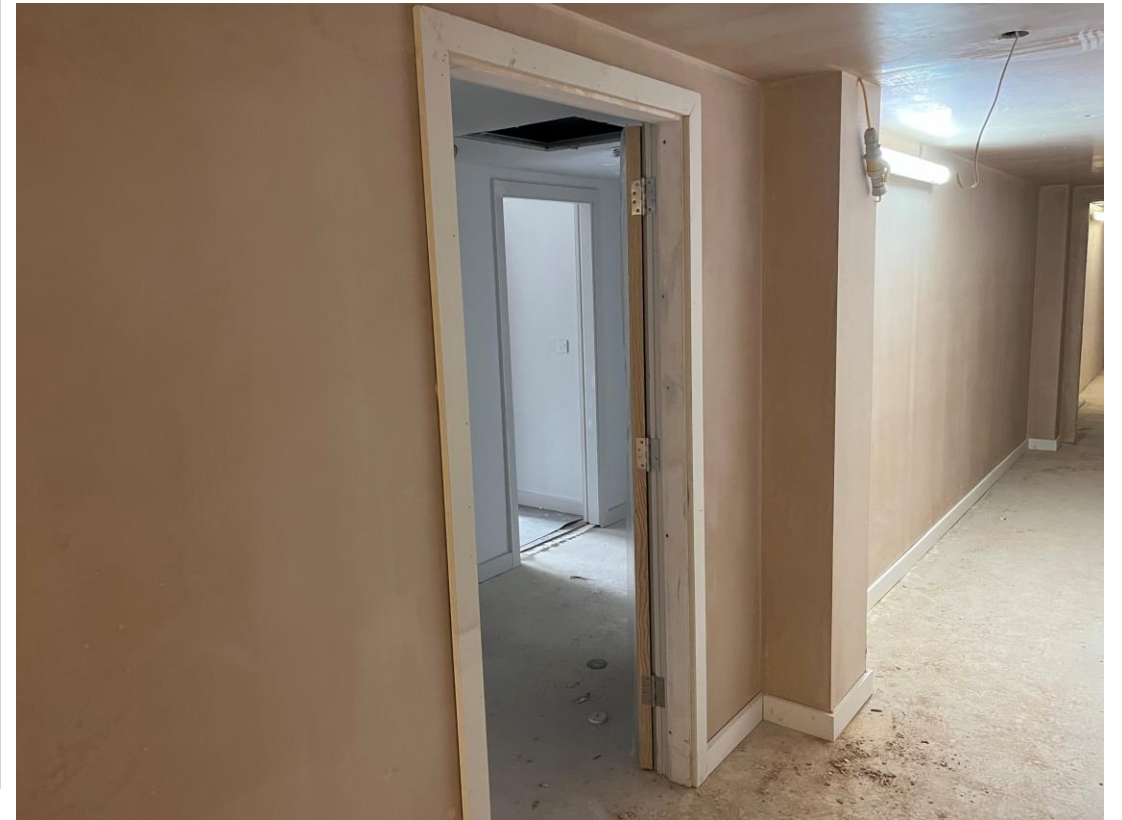
Student Wing – Internal doors, doorframes and architraves
