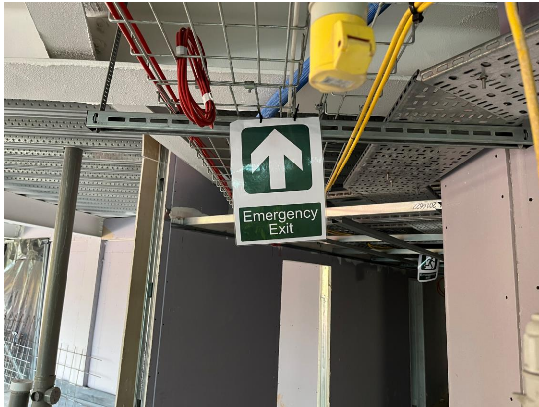
Residential Block – Fire exit signage
