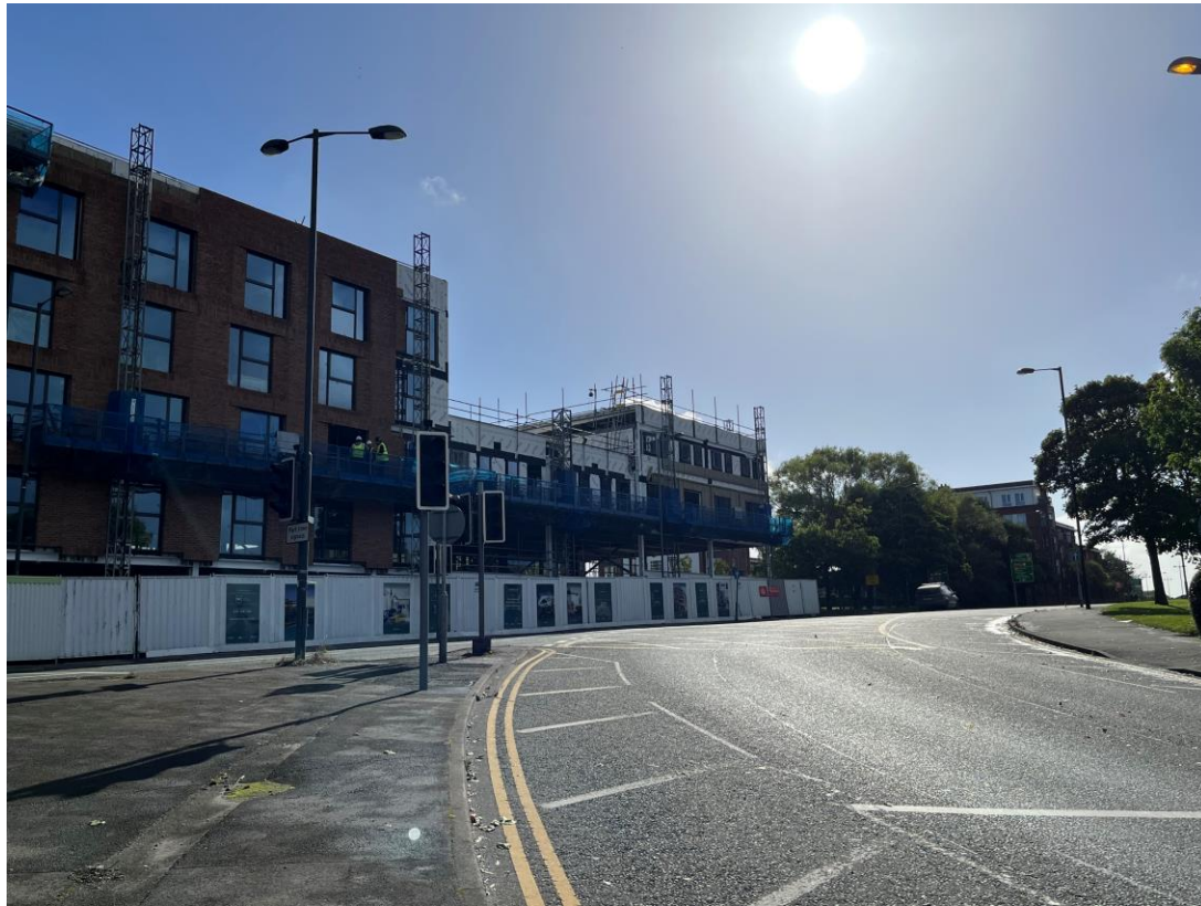
Brunswick Road - Site view
