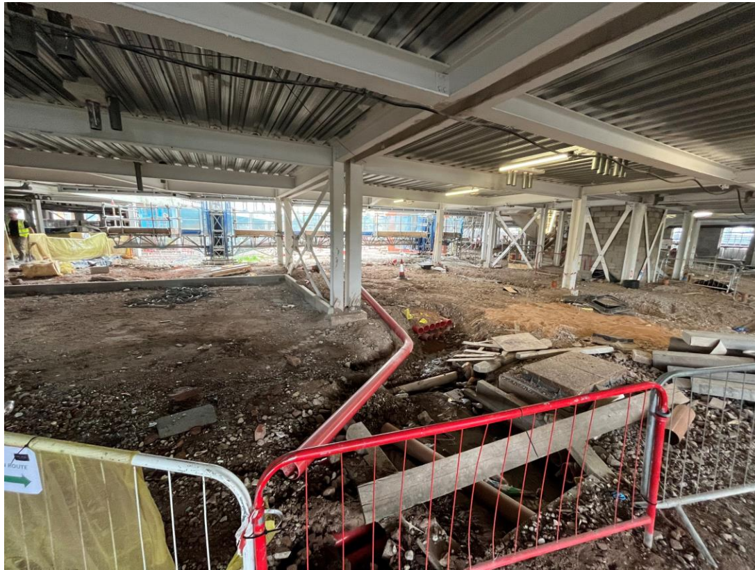
Residential Wing – Under ground drainage works on-going
