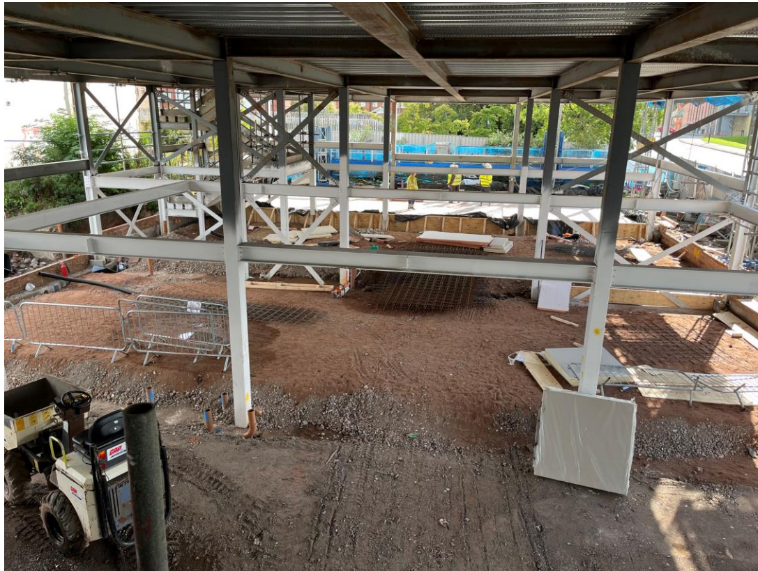
Commercial Block – Ground floor concrete slab preparations
