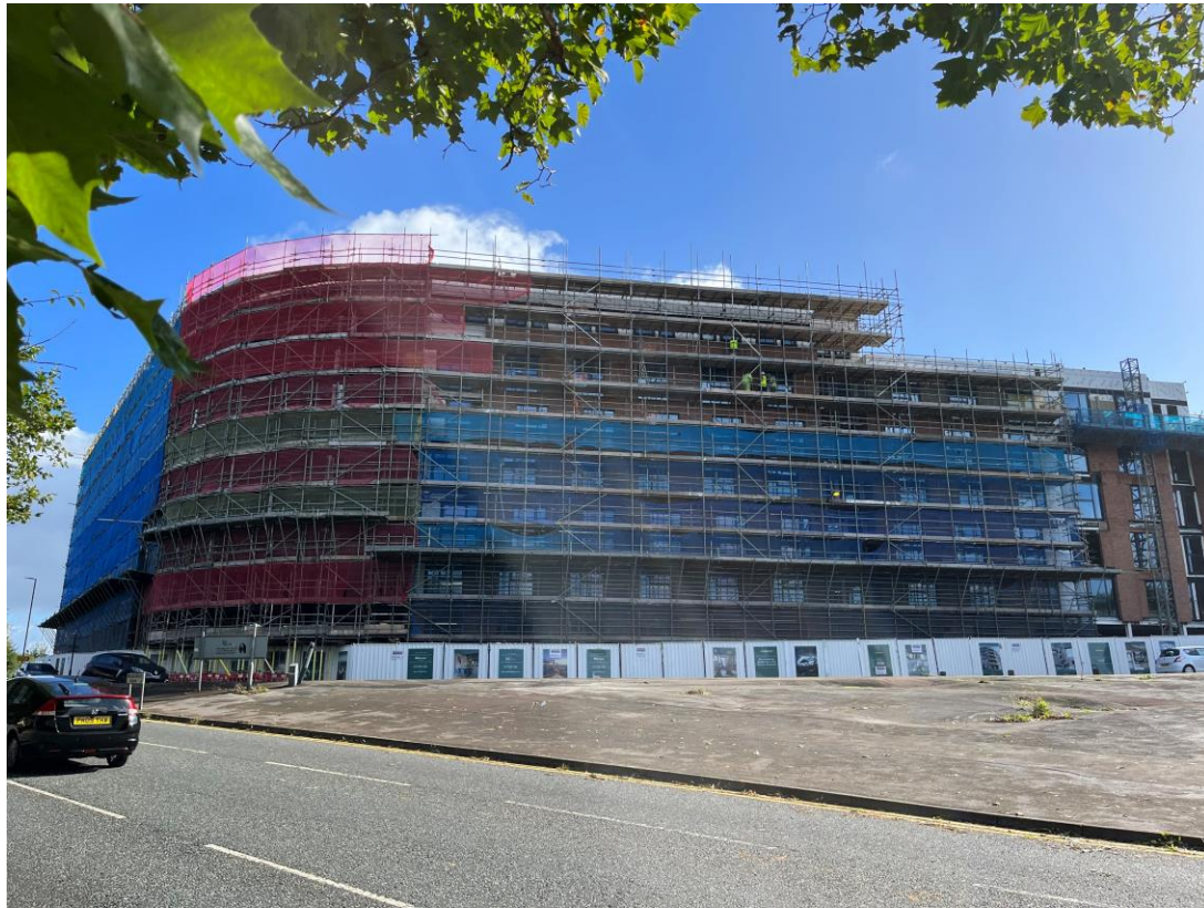
Brunswick Road - Site view
