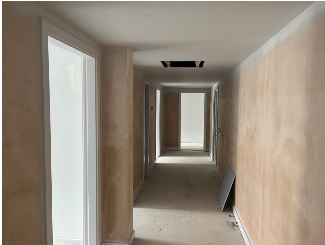
Student wing – Internal decorations on-going
