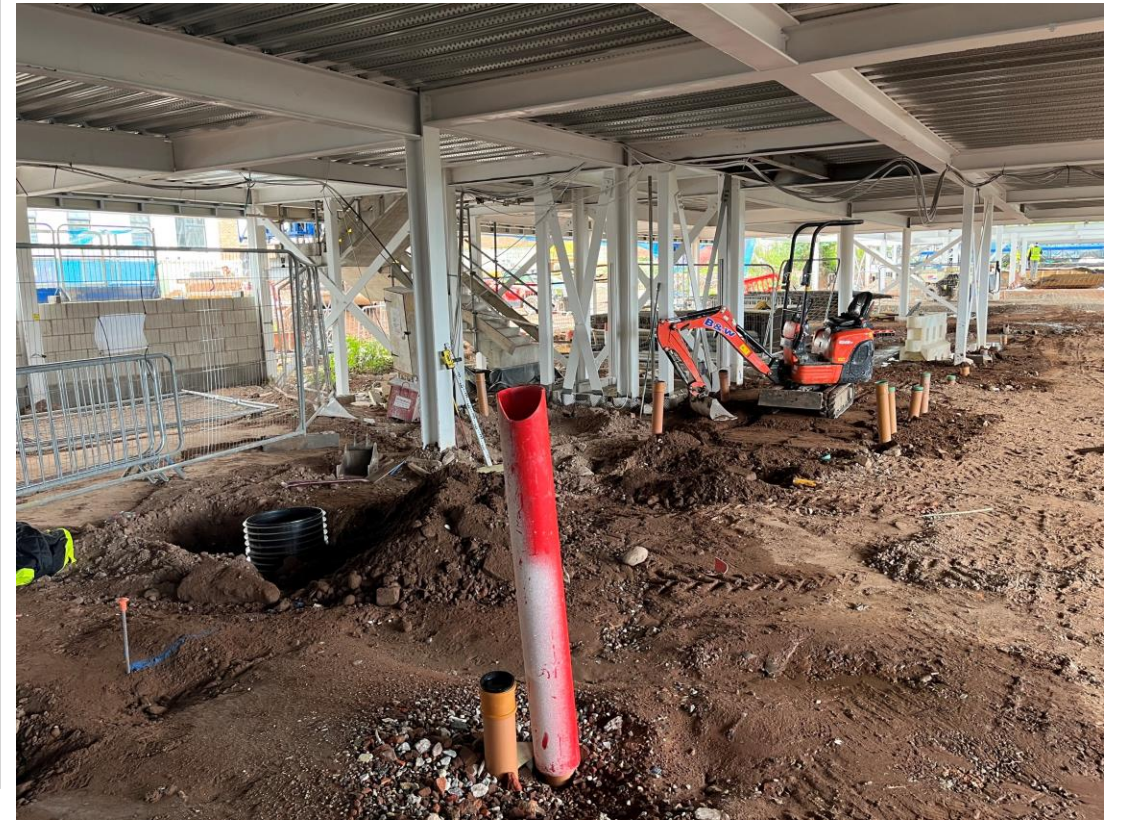
Residential Wing – Under ground drainage works on-going
