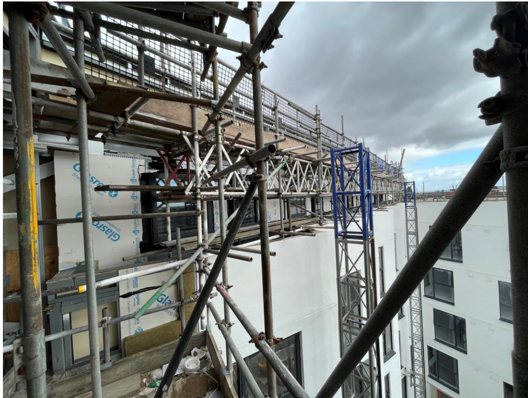
'Zig-zag' Elevation – Temporary scaffold installed
