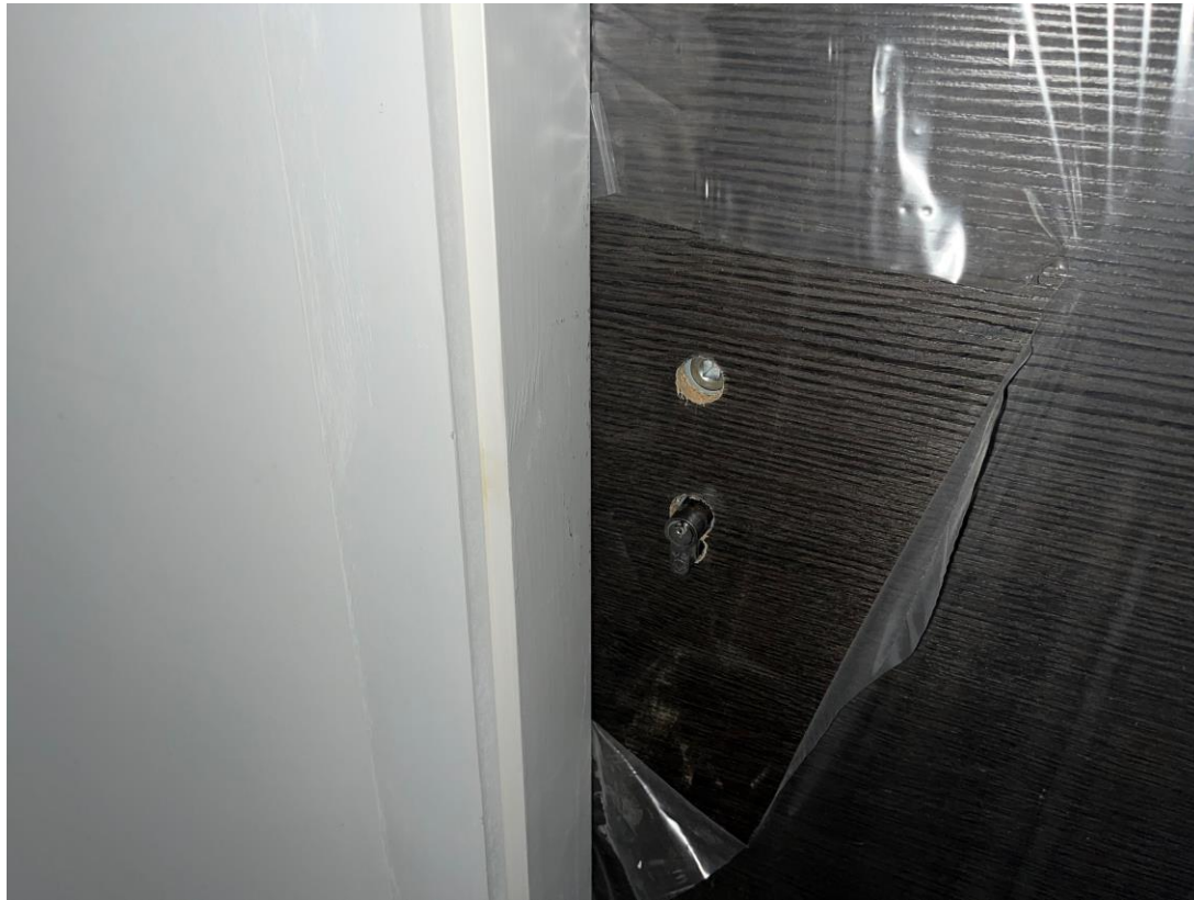
Student Wing – Door furniture commenced
