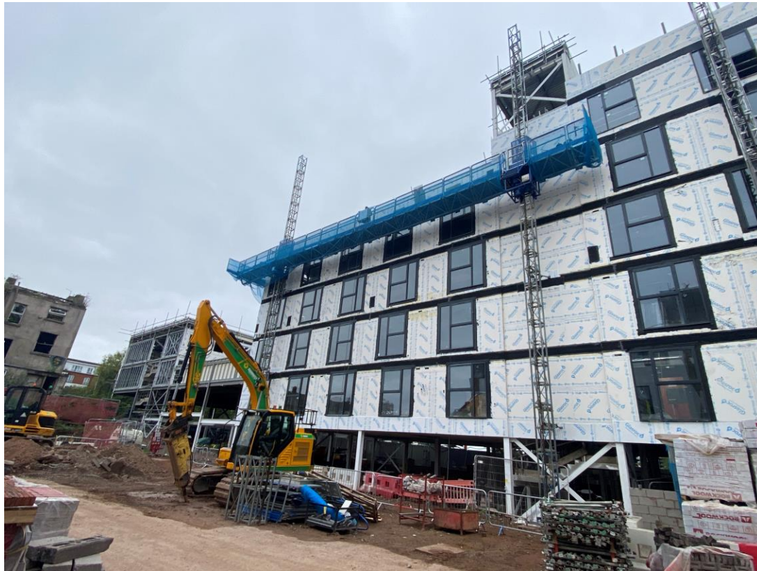
Residential Wing – SFS, weatherboard and mast climbers
