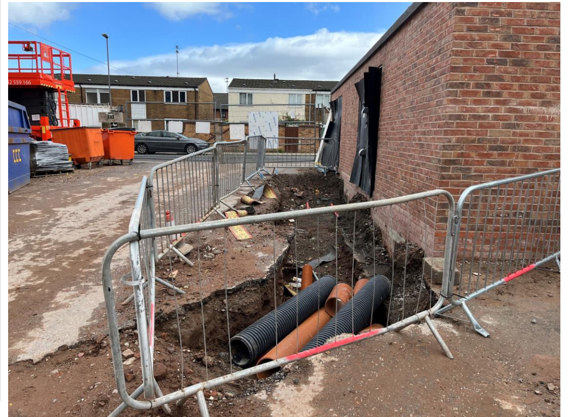
Underground drainage works on-going
