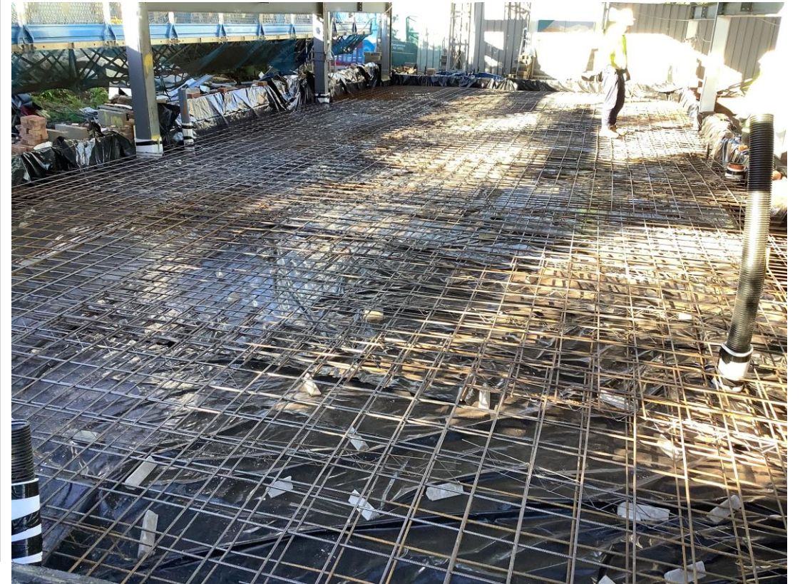
Commercial Block – Ground floor concrete slab preparations
