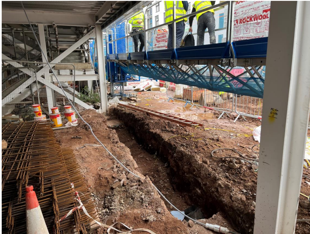
Commercial Block – External wall foundations on-going
