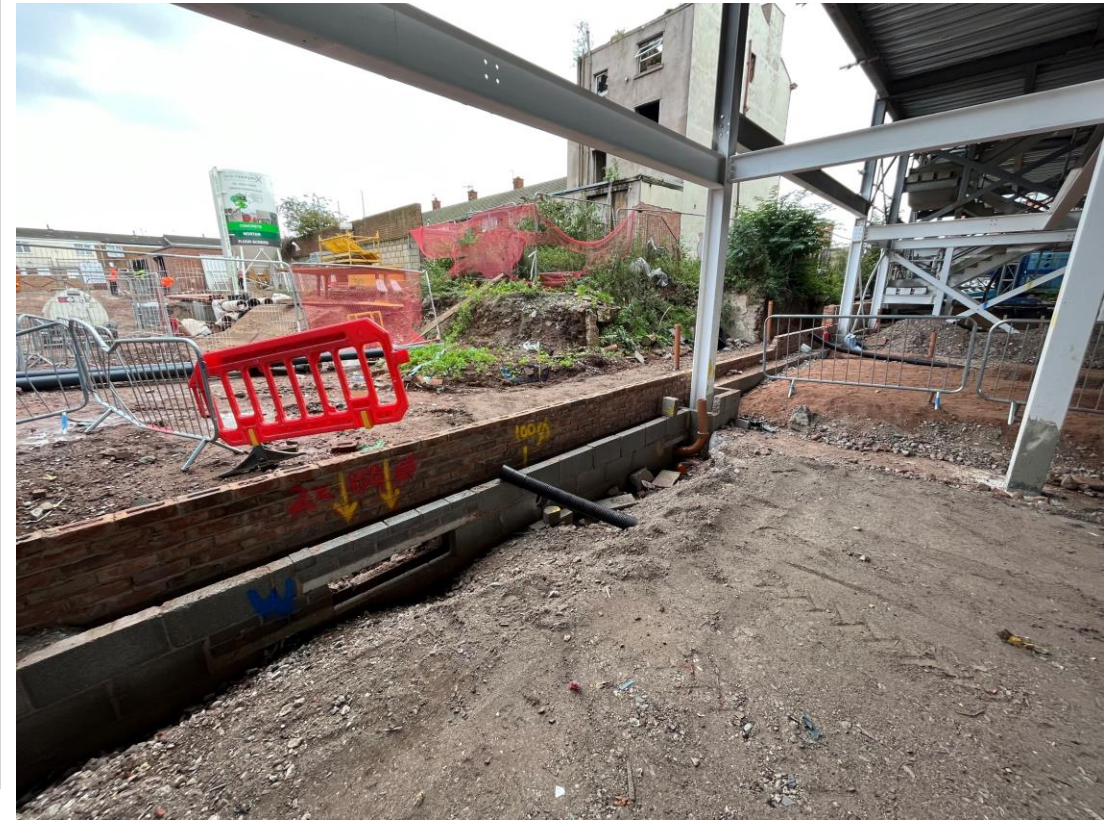
Commercial Block - Retaining wall complete
