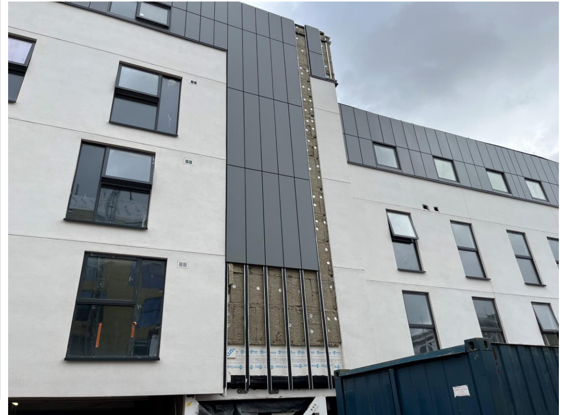
Student wing – Cladding progress
