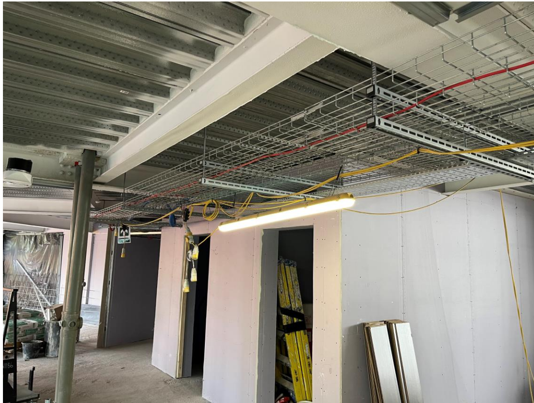
Residential Wing – Cable trays on-going
