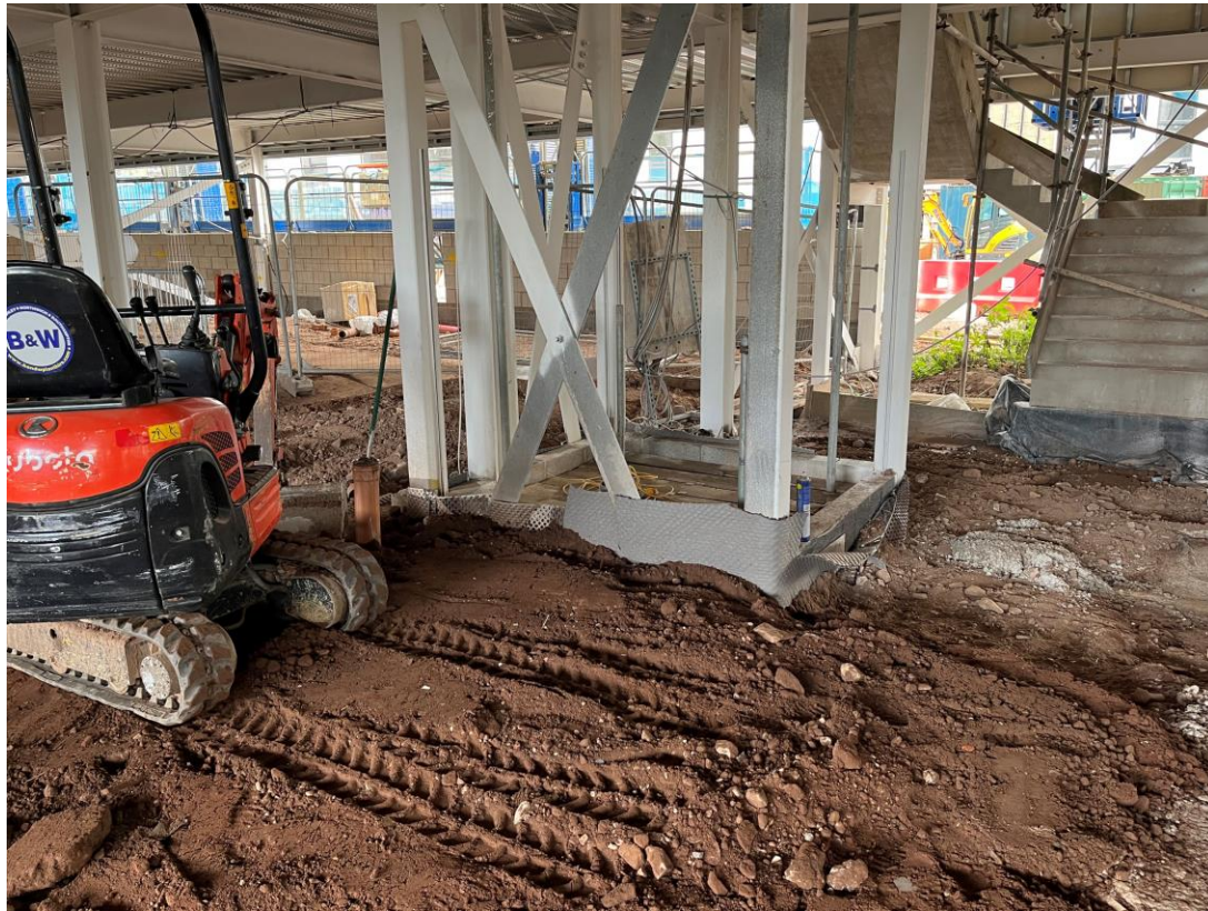
Residential Wing - Lift core tanking complete
