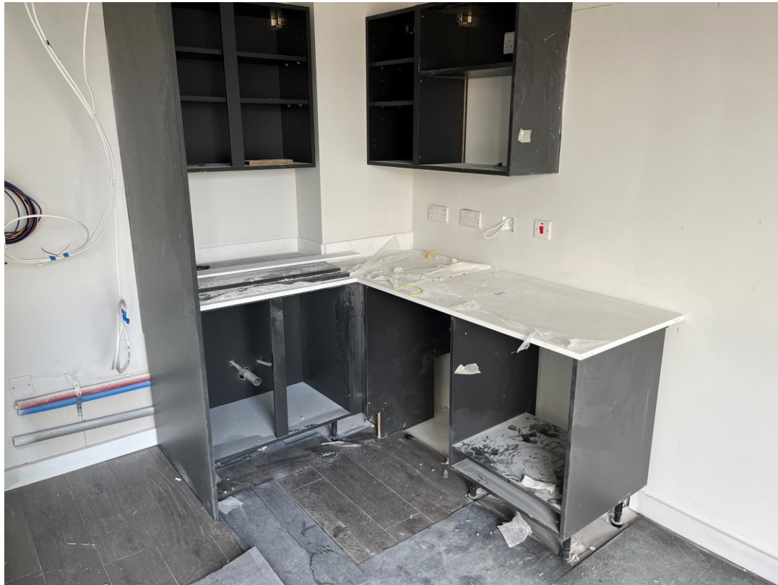
Student Wing – Kitchen units on-going
