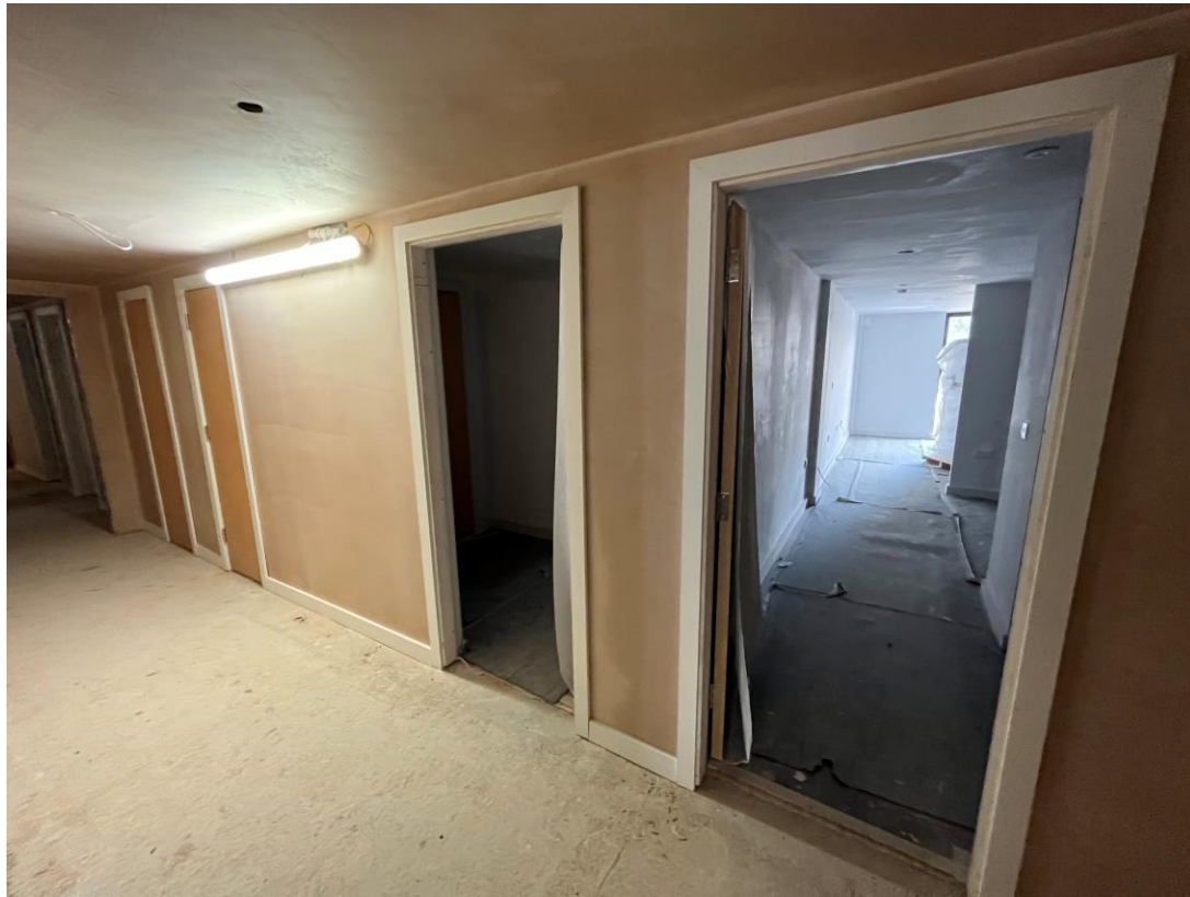
Student Wing – Internal doors, doorframes and architraves
