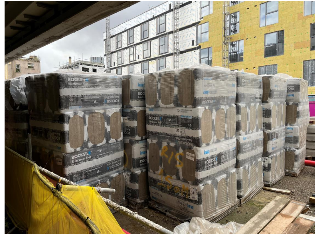
Material storage – Rocksil Insulation
