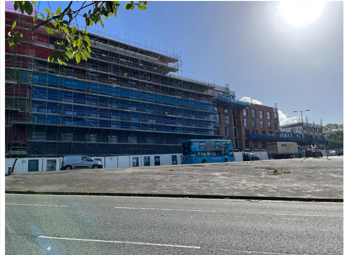
Brunswick Road - Site view
