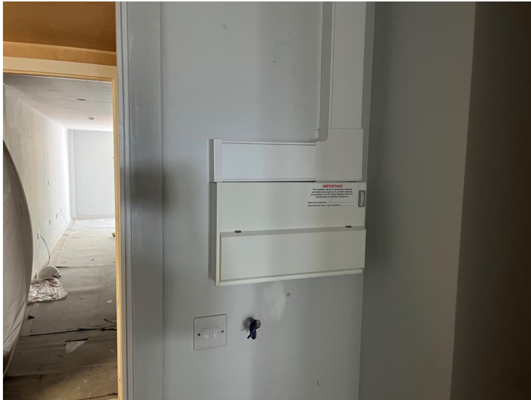
Student Wing – Electrical consumer units on-going
