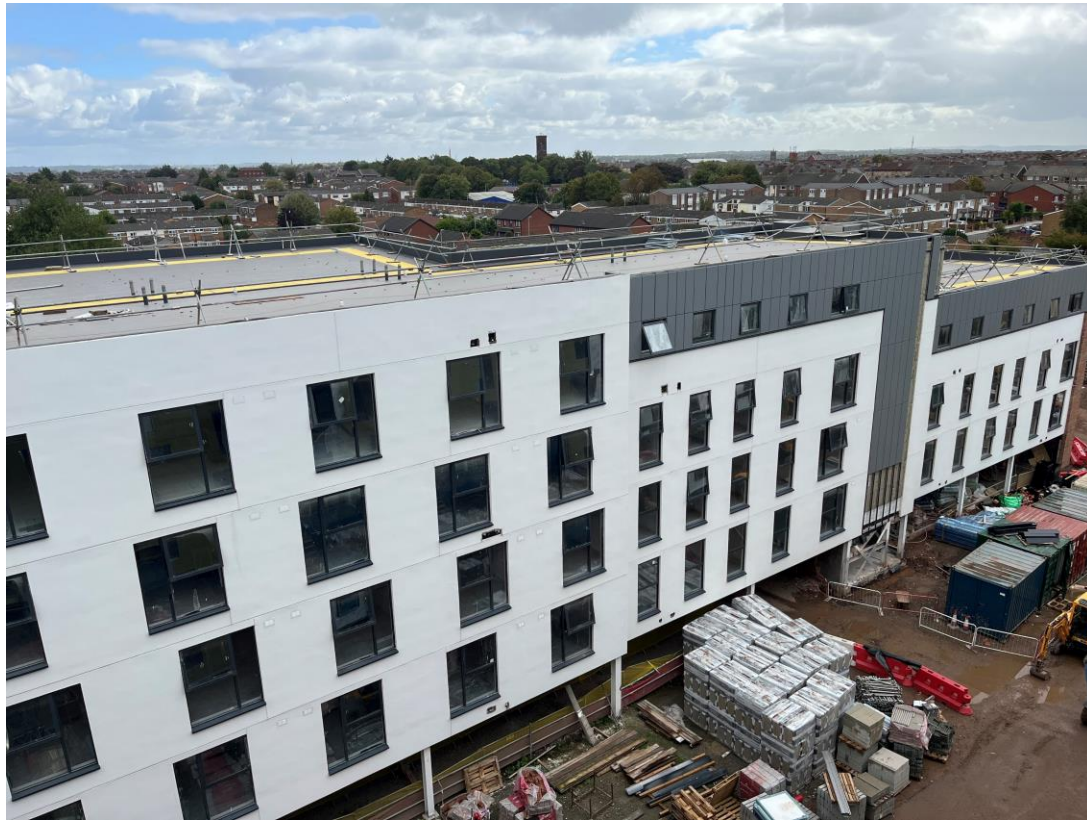
Student Wing – Cladding progress
