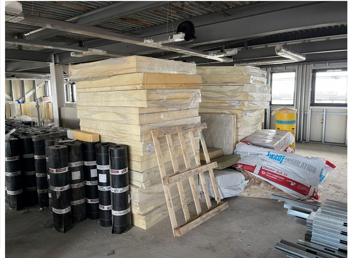
Material storage – Insulation and roofing materials
