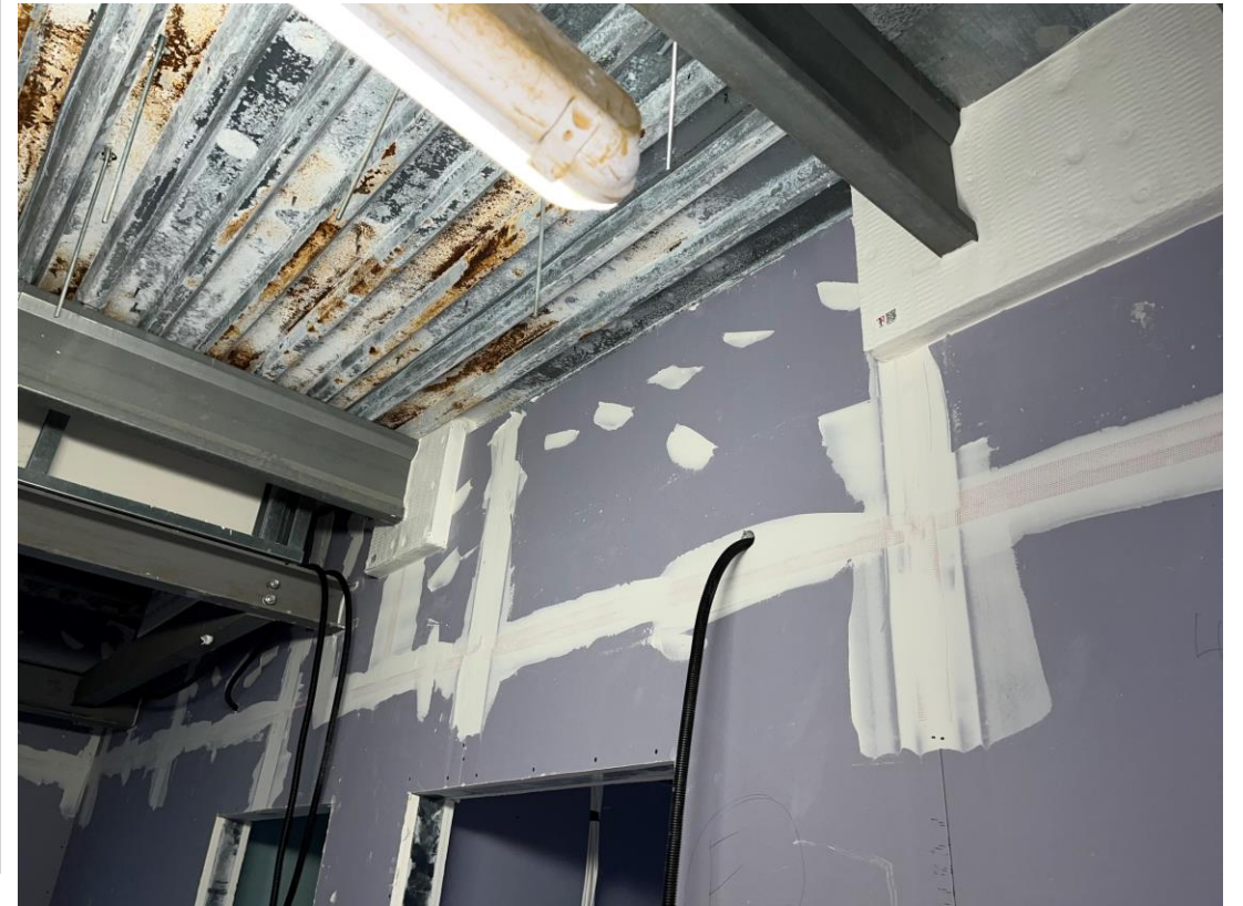
Student Wing – Fire stopping works to upper floors on-going
