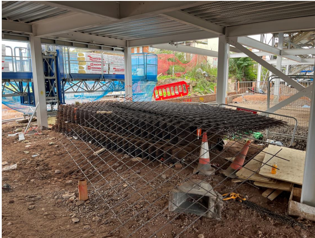
Material storage – Steel reinforcement
