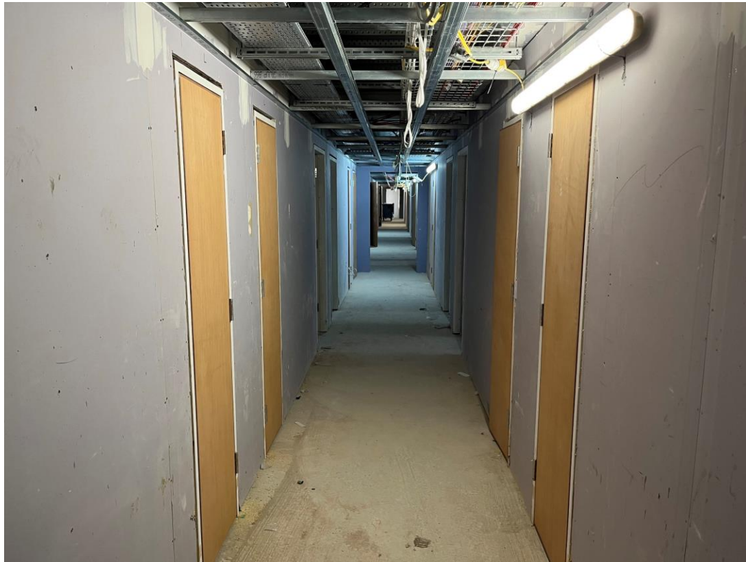
Student Wing – Internal doors to maintenance cupboards
