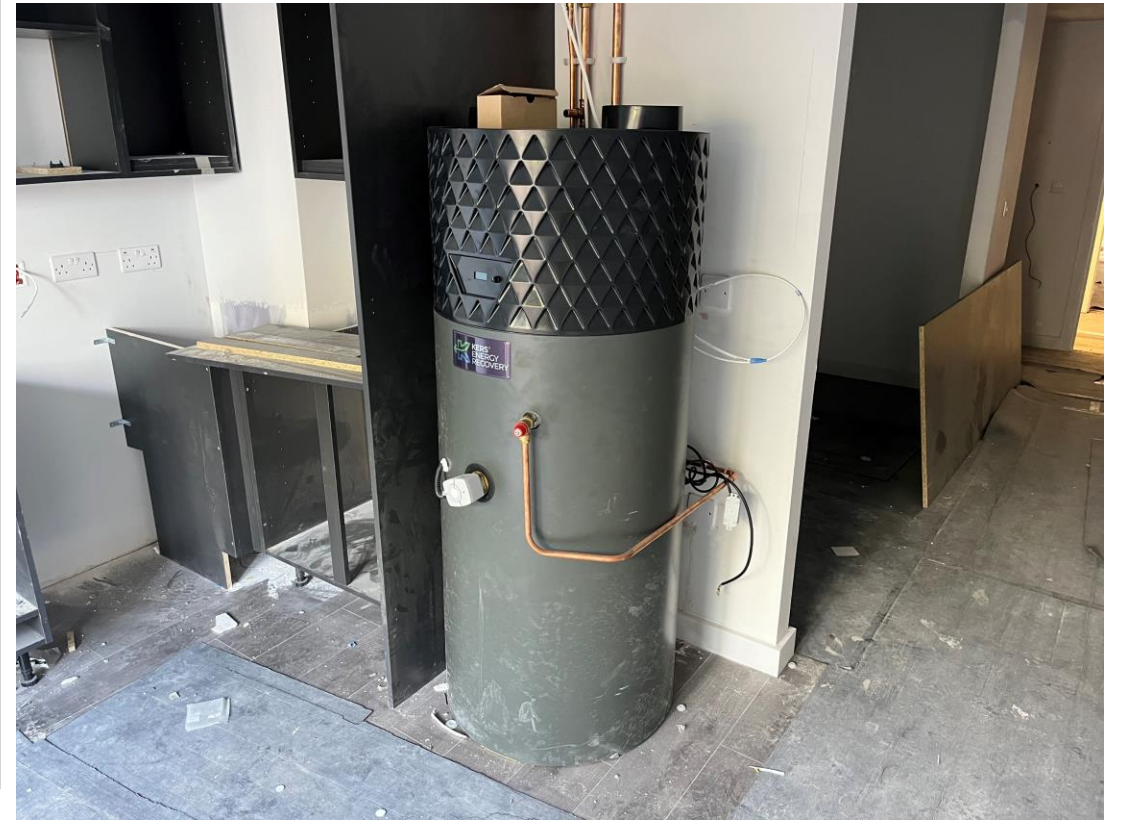
Student Wing – KERS Units installation commenced
