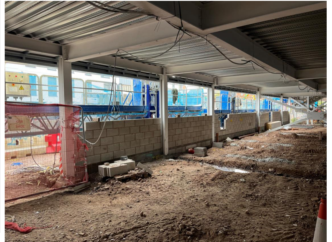
Residential Block – External wall blockwork on-going
