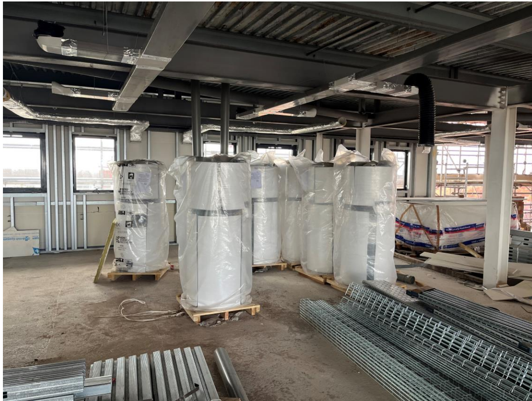
Material storage – KERS units
