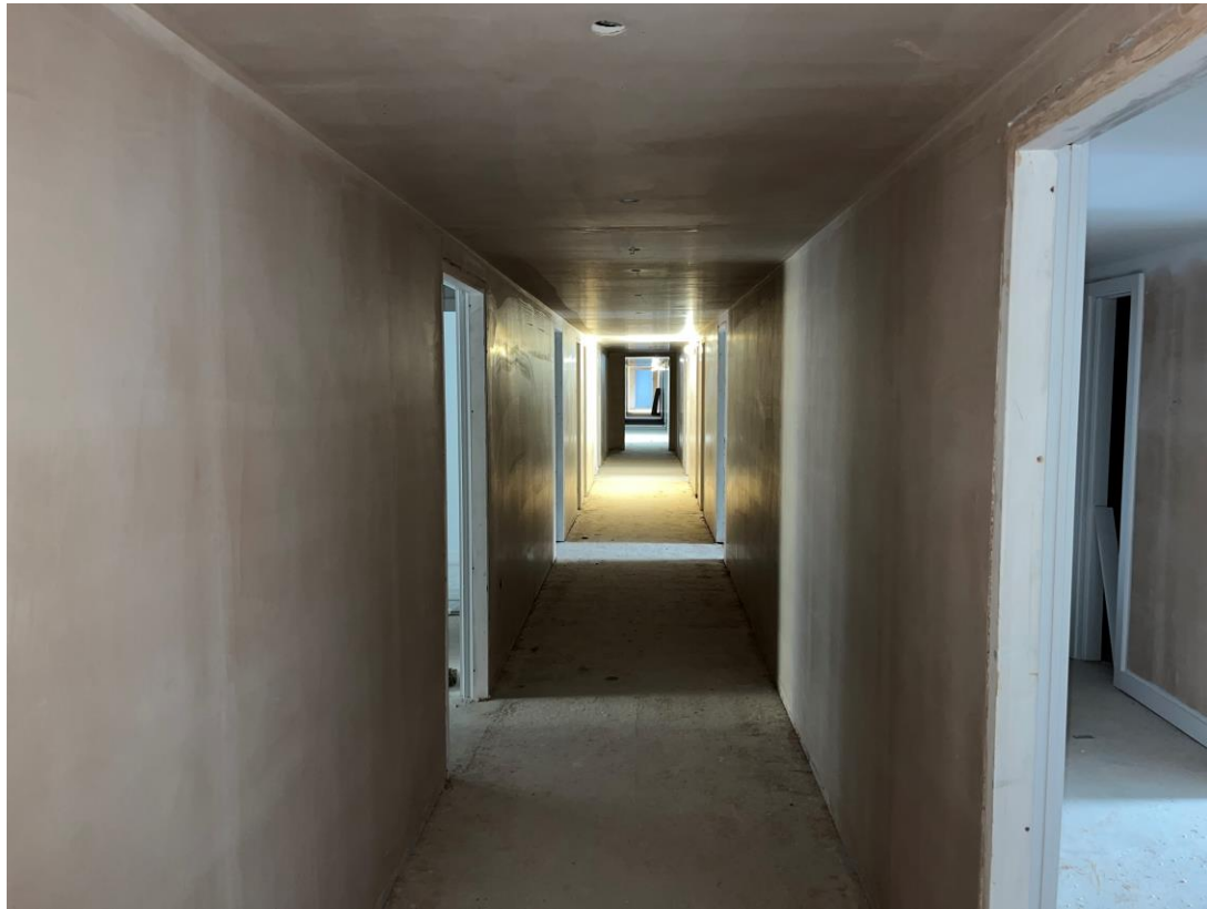
Student Wing – Plaster to circulation areas
