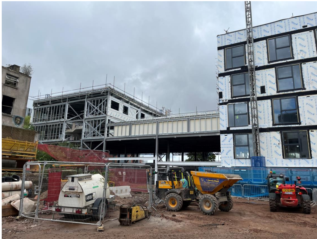
Commercial Block – SFS, weatherboard and mast climbers
