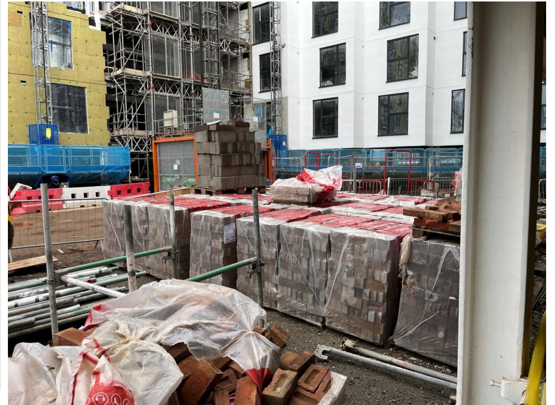
Material storage – Red brick and industrial block
