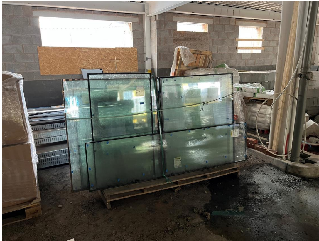
Material storage – Glazing panels
