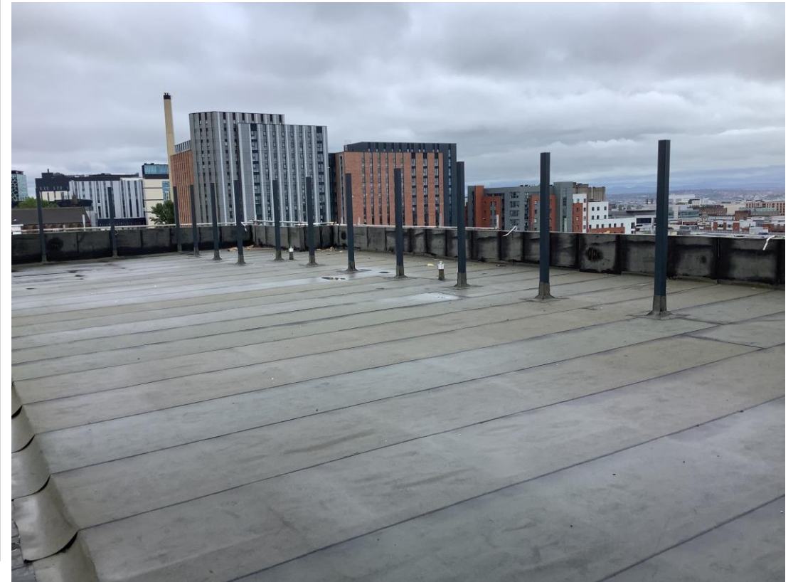
Commercial Block – External metal balustrade
