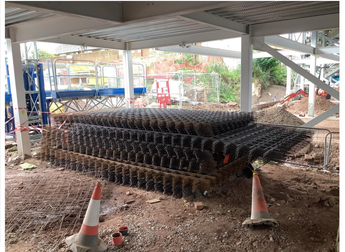
Material storage – Steel reinforcement
