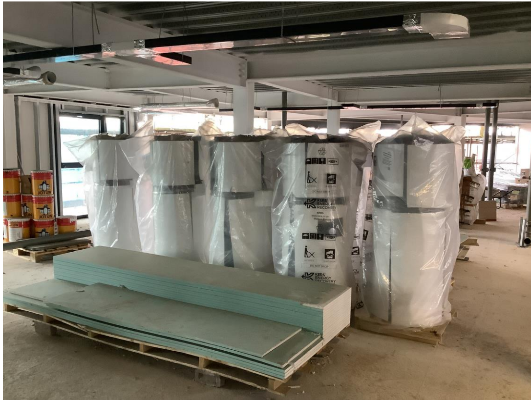
Material storage – KERS units
