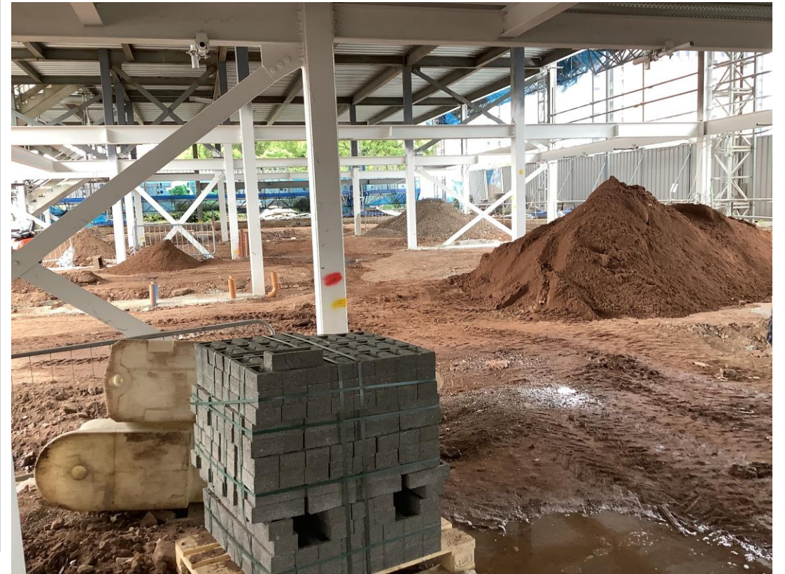
Commercial Block - Ground infill and site levelling
