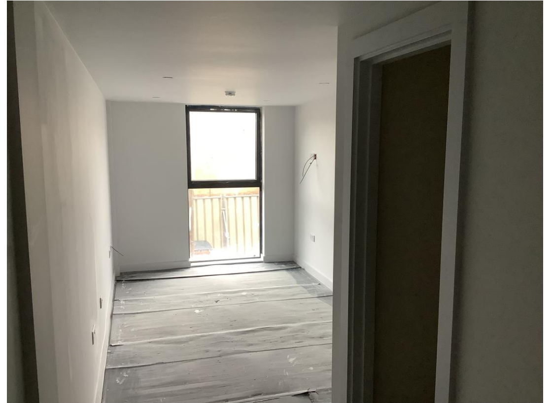
Student wing – Internal finishes and decorations
