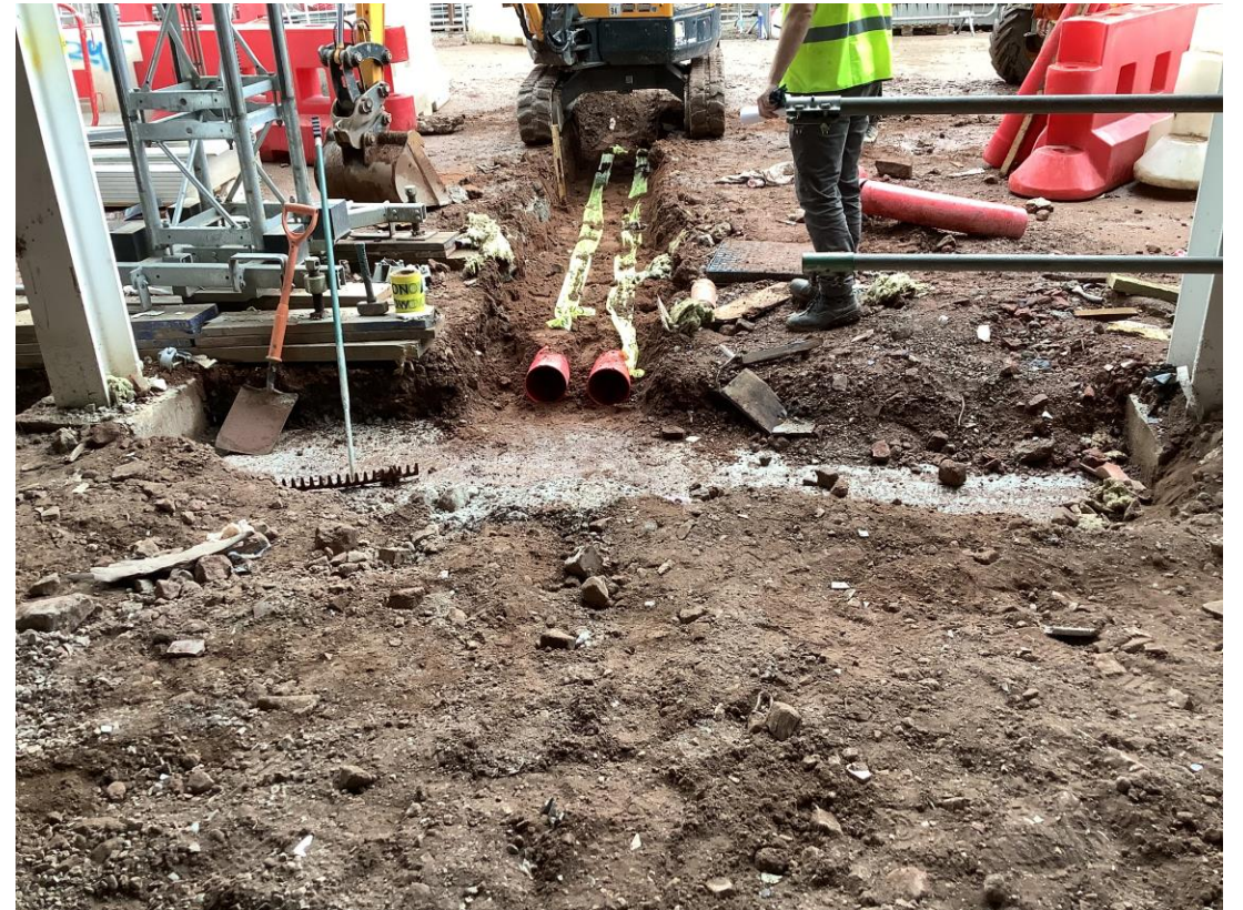
Residential Wing – Under ground drainage works
