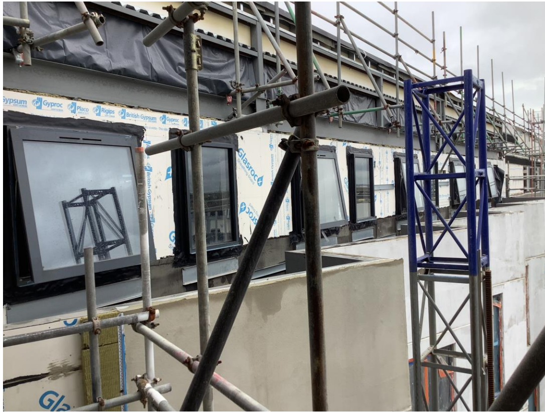
'Zig-zag' Elevation – Windows & render progress
