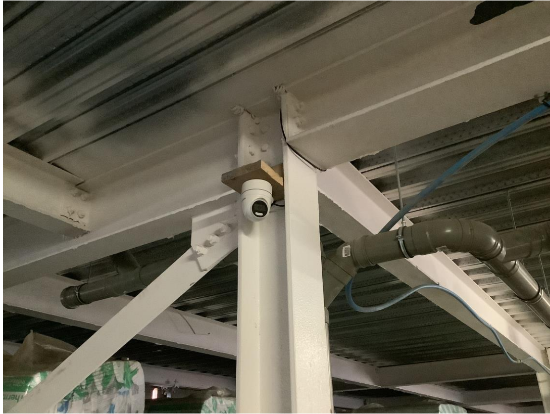
Student Wing – Installation of CCTV to undercroft parking area
