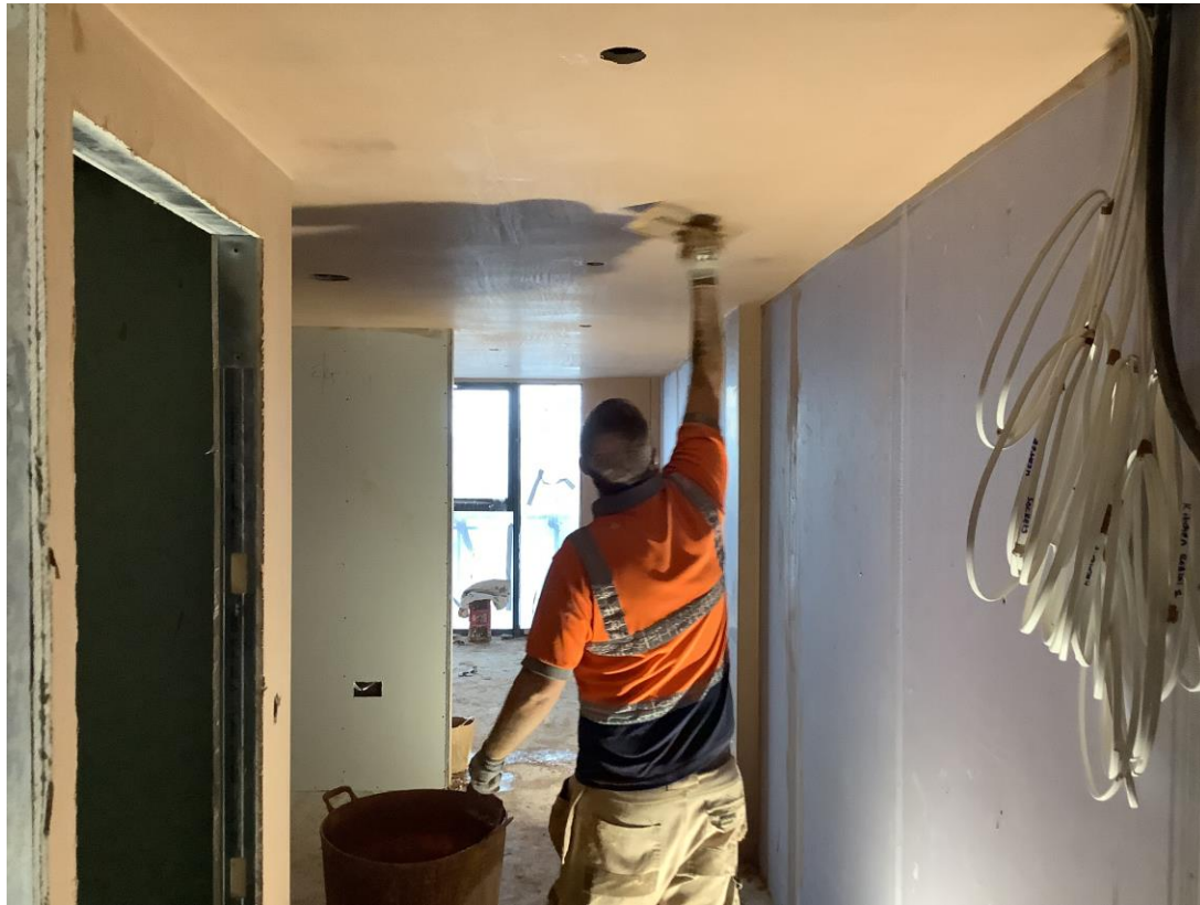
Residential Wing – Studio walls & ceilings being skimmed
