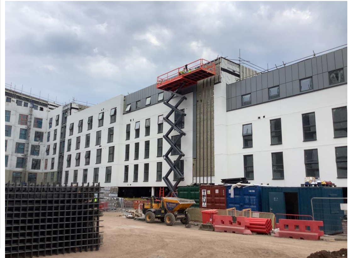
Student wing – MEWP & cladding progress
