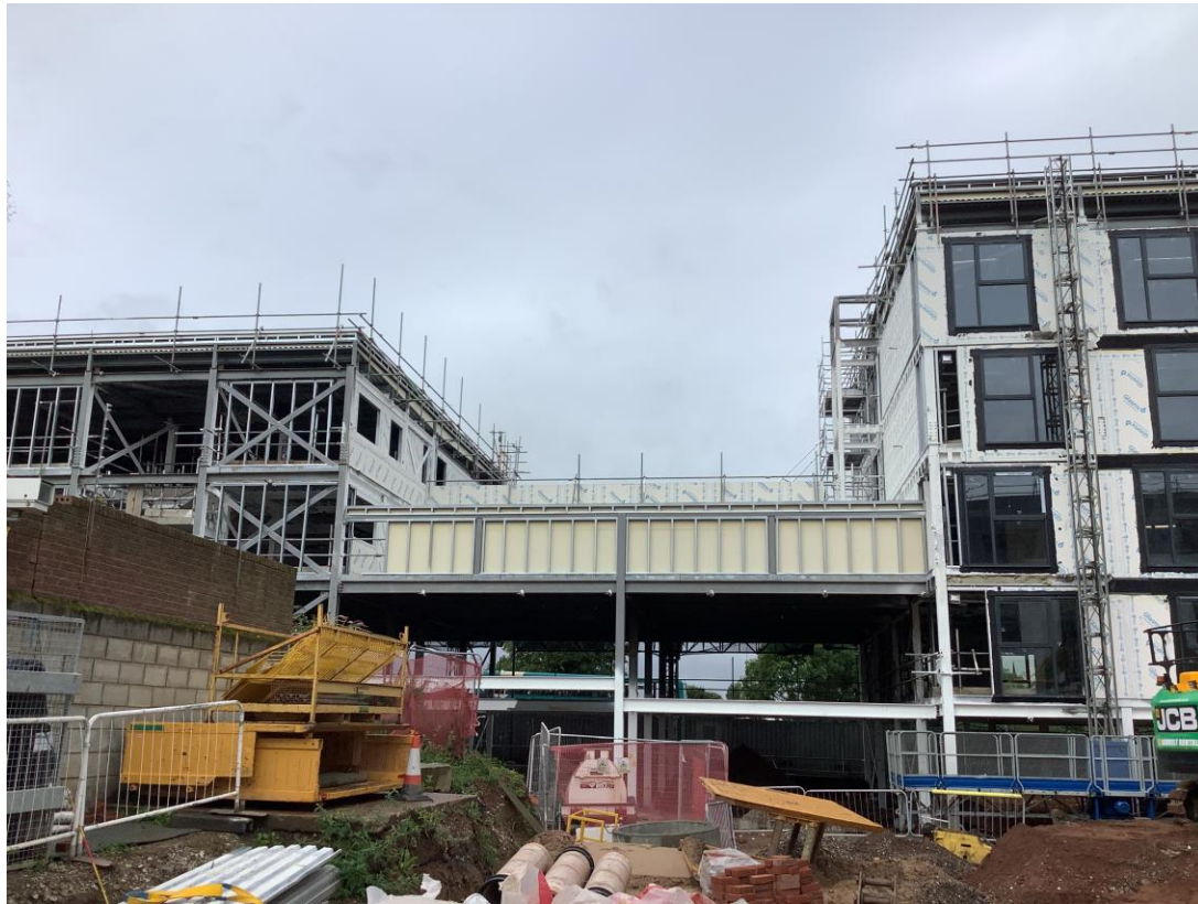
Commercial Block – SFS, weatherboard and windows
