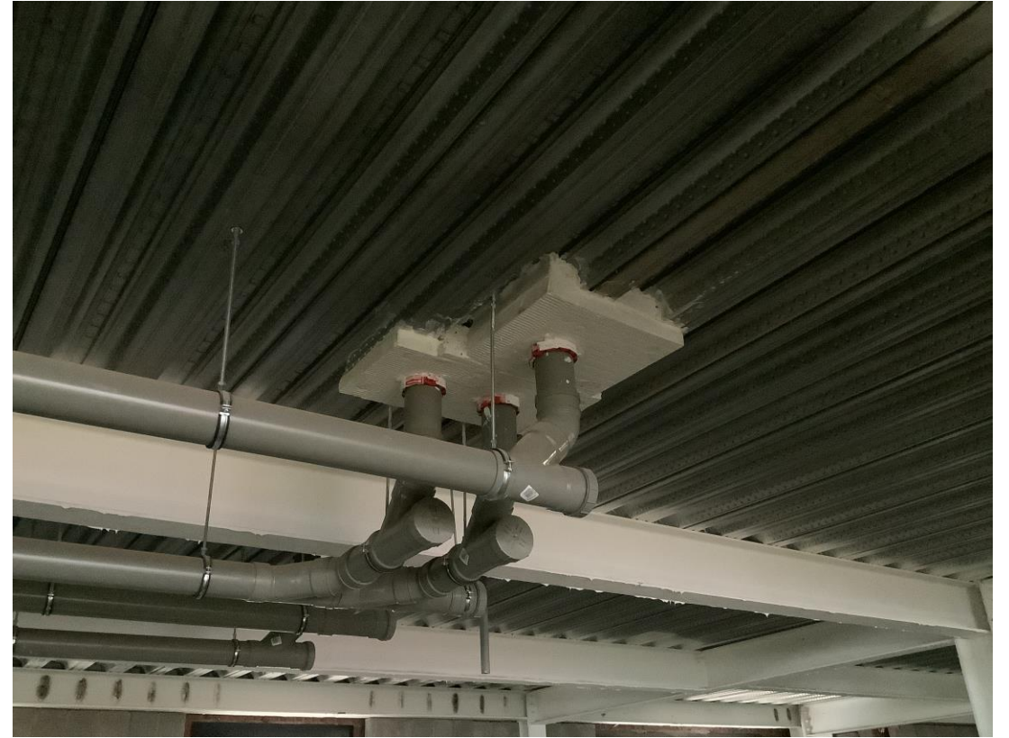
Student Wing – Fire stopping works
