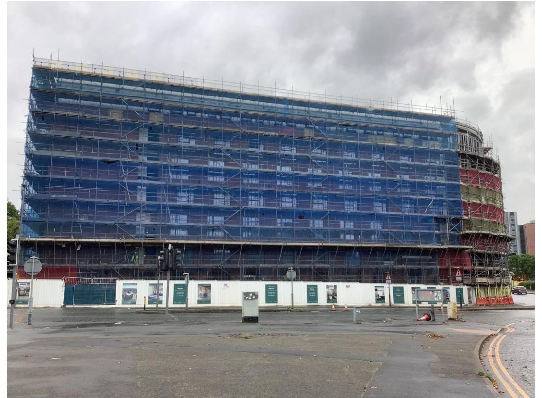
West Derby Road - Site view
