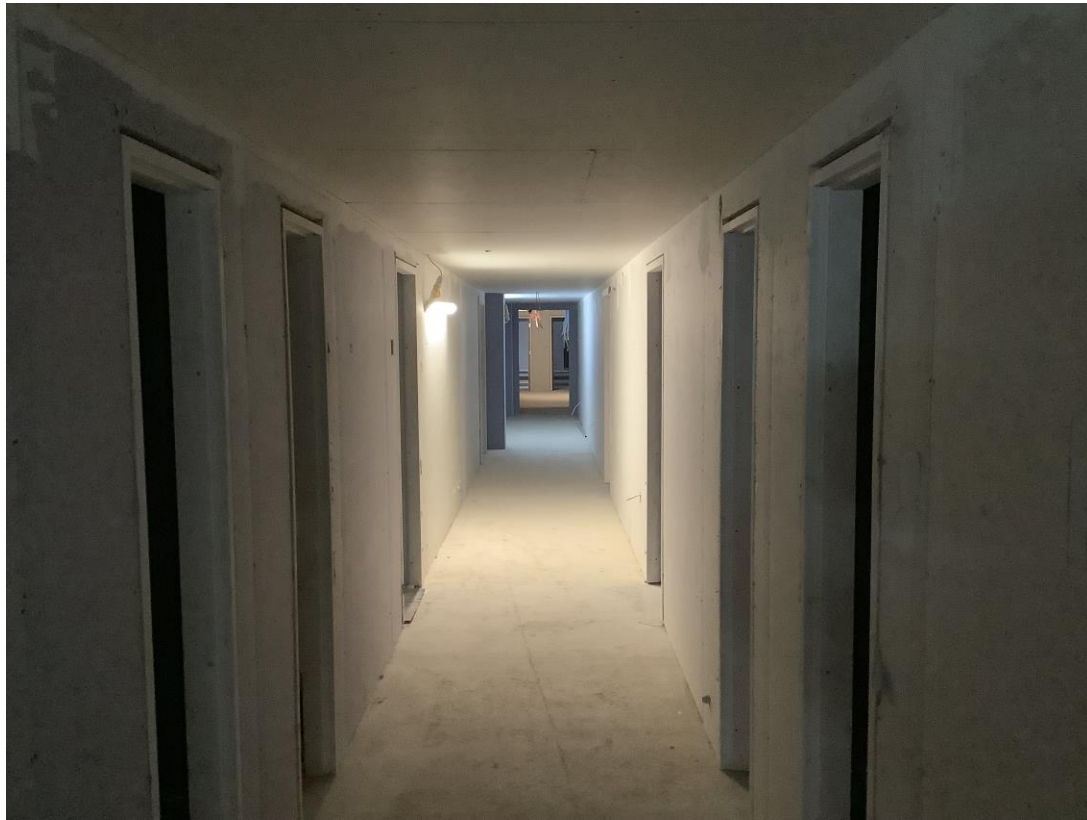
Student Wing – Internal doorframes and boarding of ceilings & partitions
