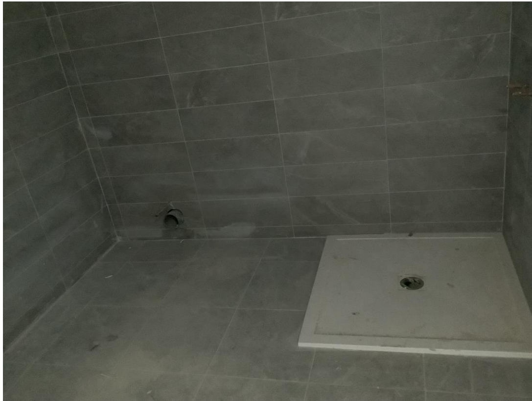
Student Wing - Bathroom tiles and shower tray
