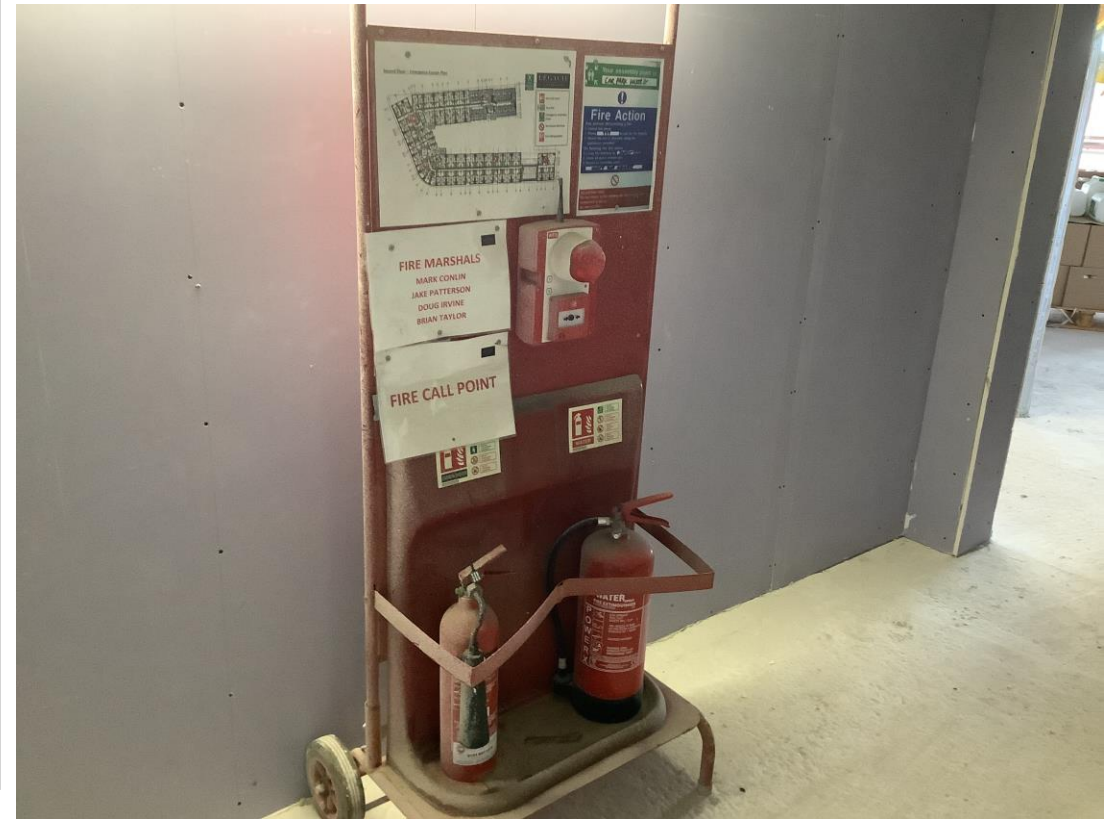
Residential Block – Fire call point
