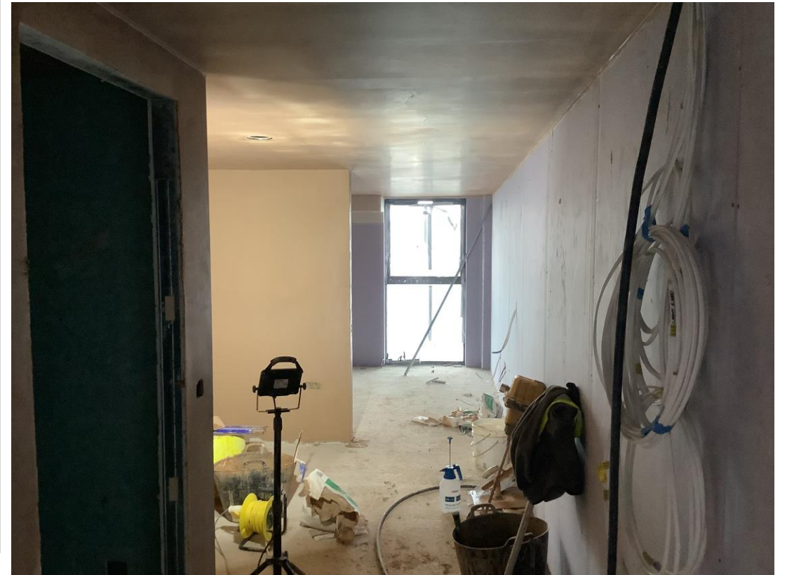
Residential Wing – Studio walls & ceilings being skimmed
