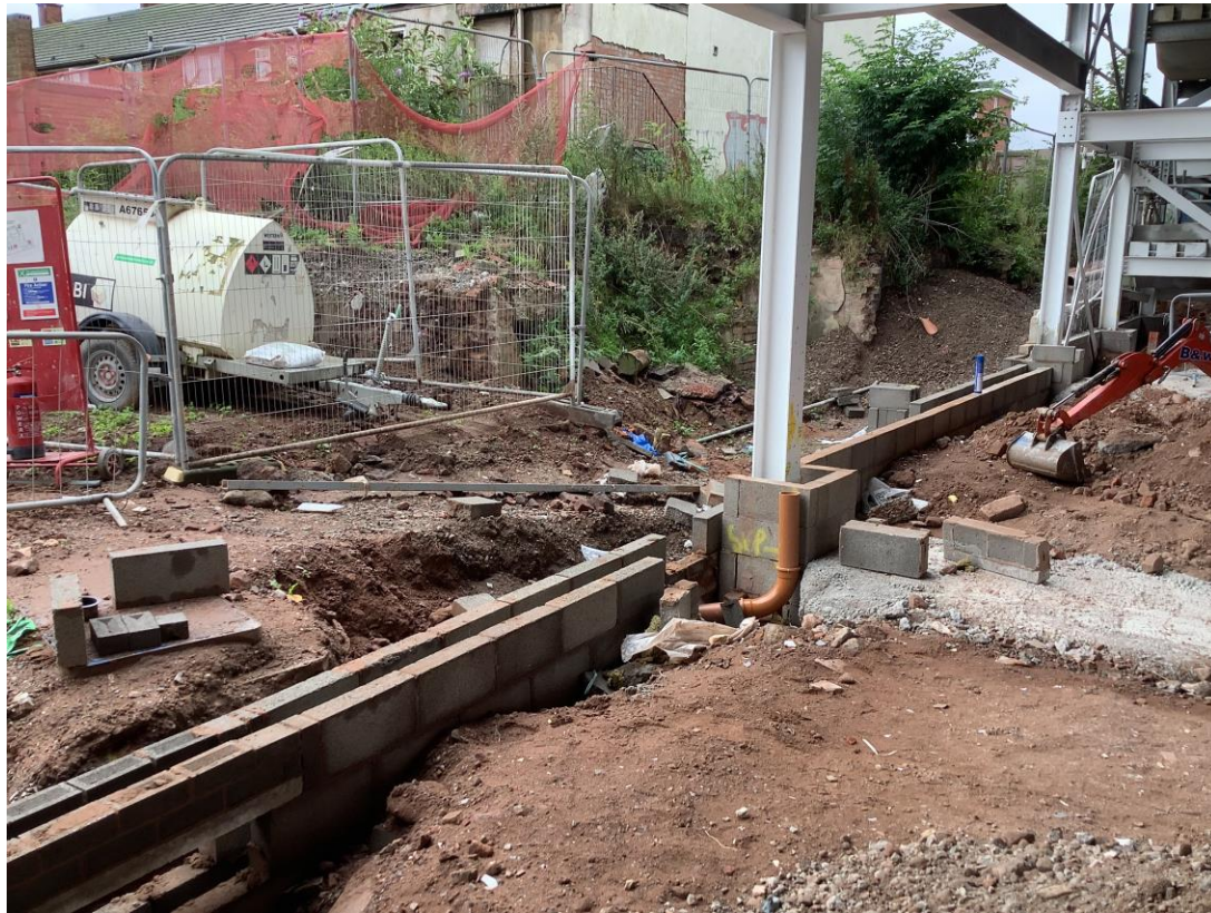
Commercial Block - Retaining wall on-going
