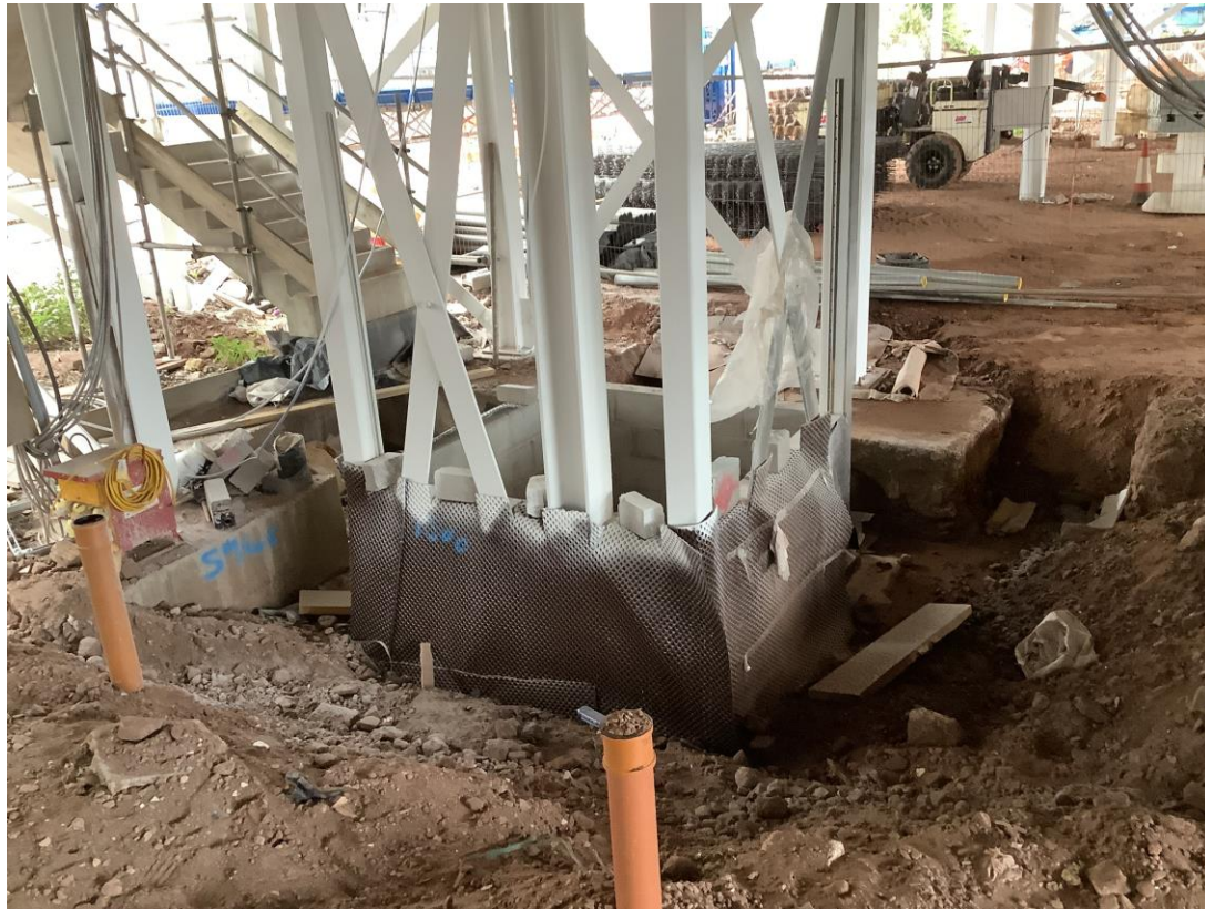
Residential Wing - Lift core tanking
