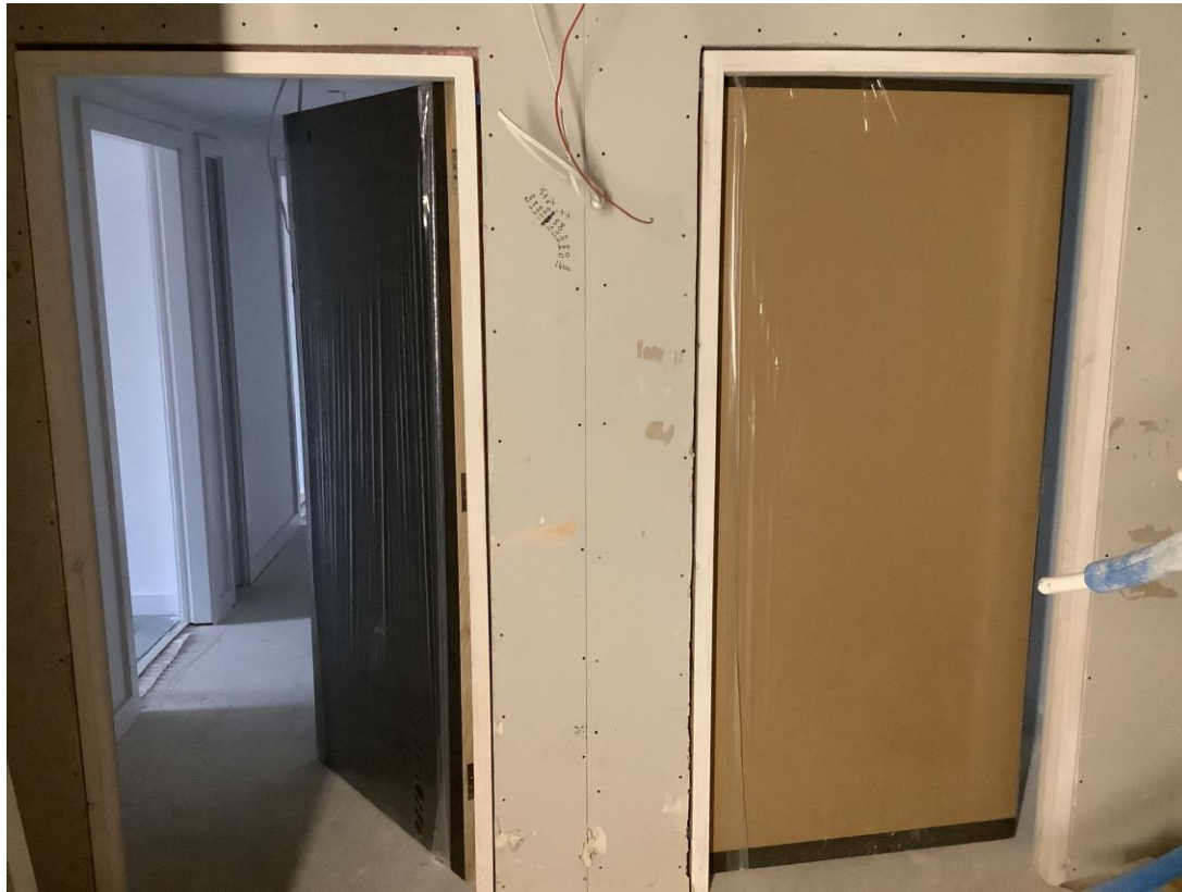
Student Wing – Cluster room doors installed and protected
