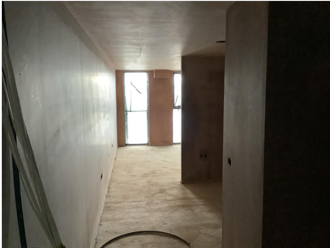
Residential Block – Studio walls boarded & skimmed
