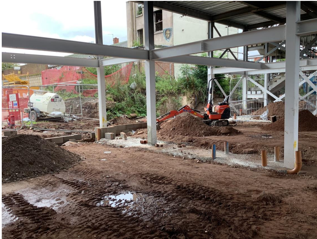
Commercial Block – Under ground drainage & site levelling works
