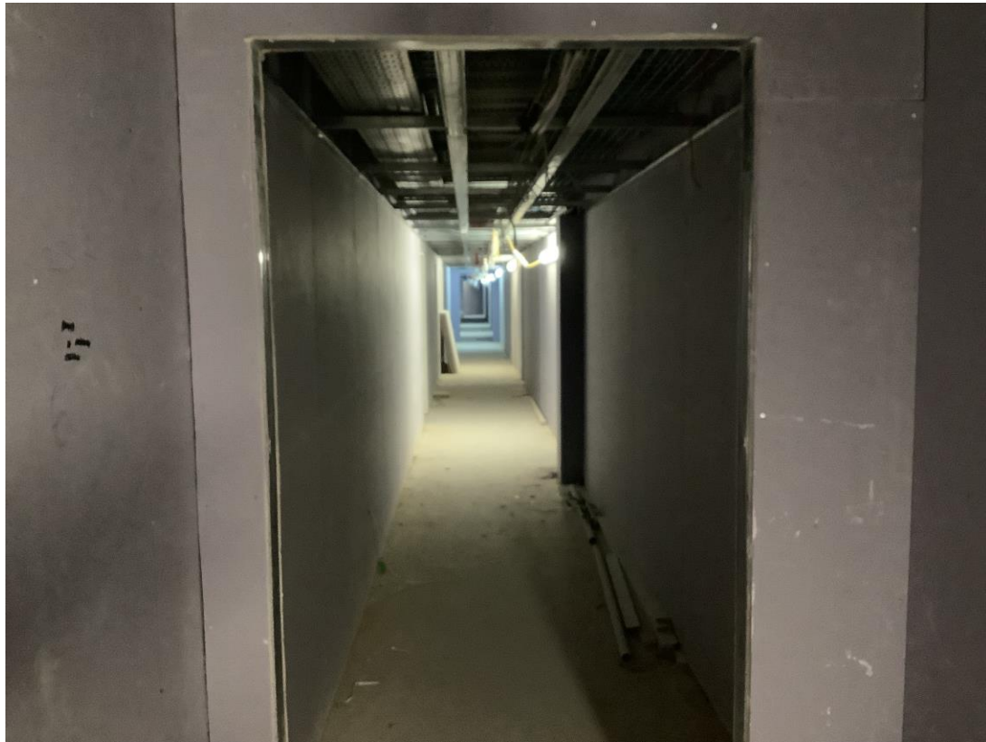
Residential Wing – Boarding of partitions to circulation areas
