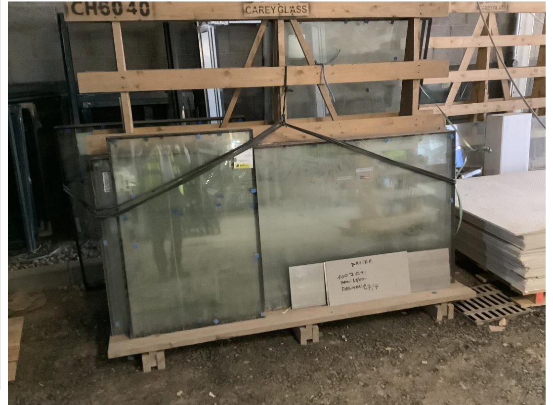
Material storage – Glazing panels
