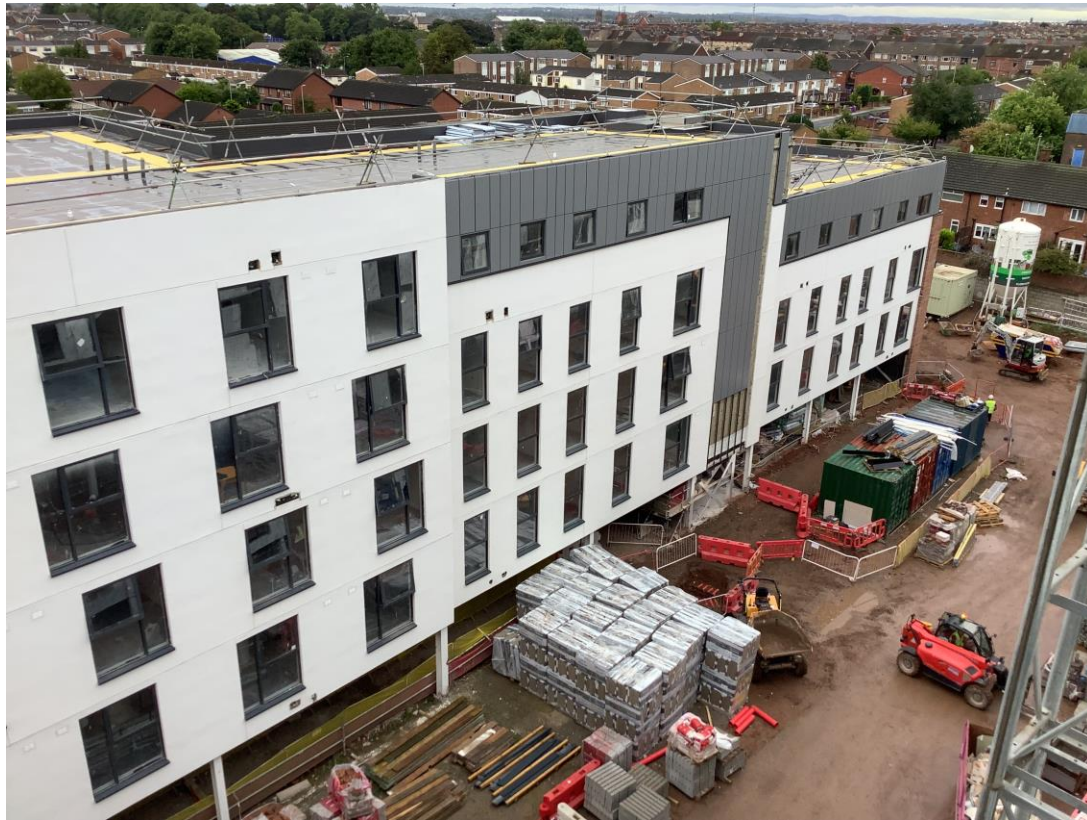
Student Wing – Cladding progress
