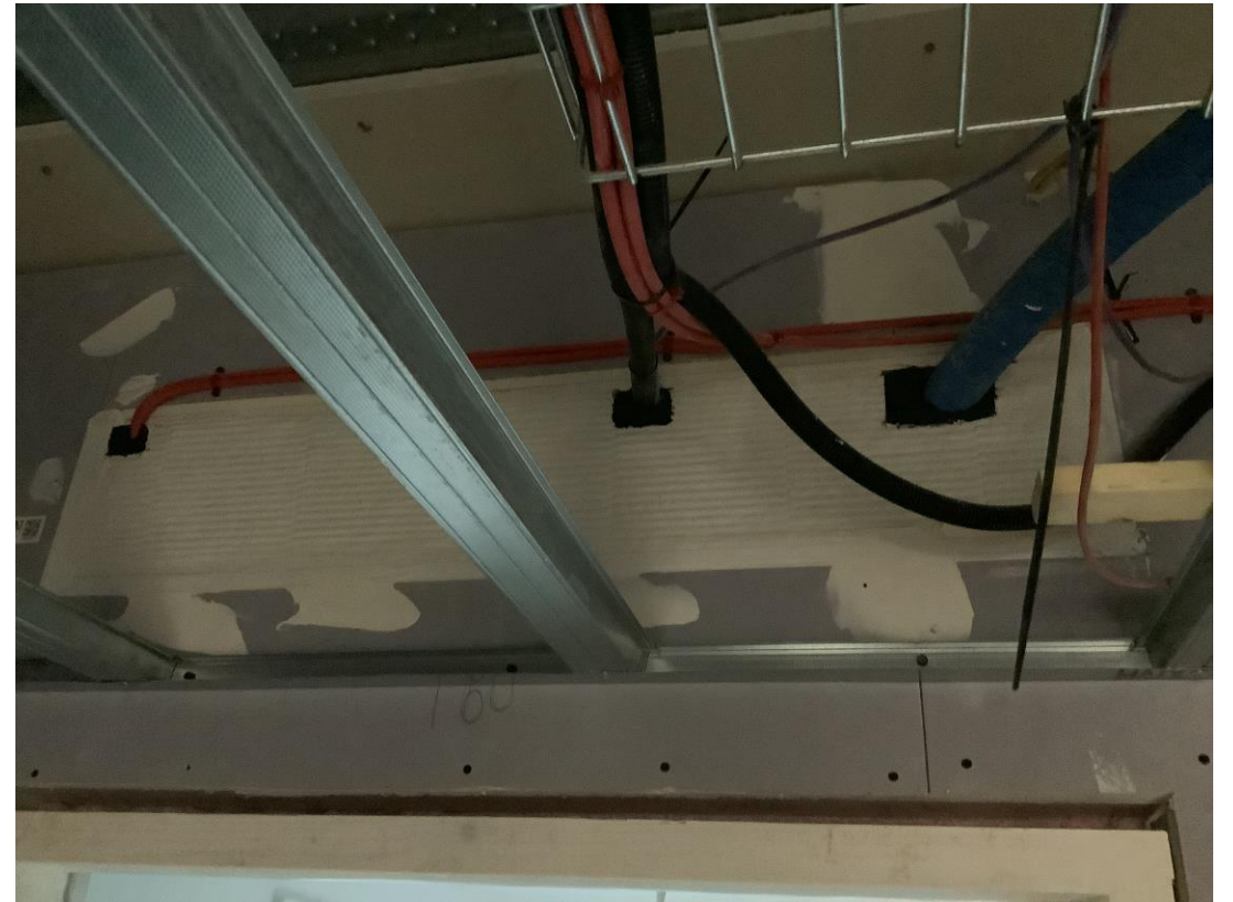
Residential Wing - Fire stopping works
