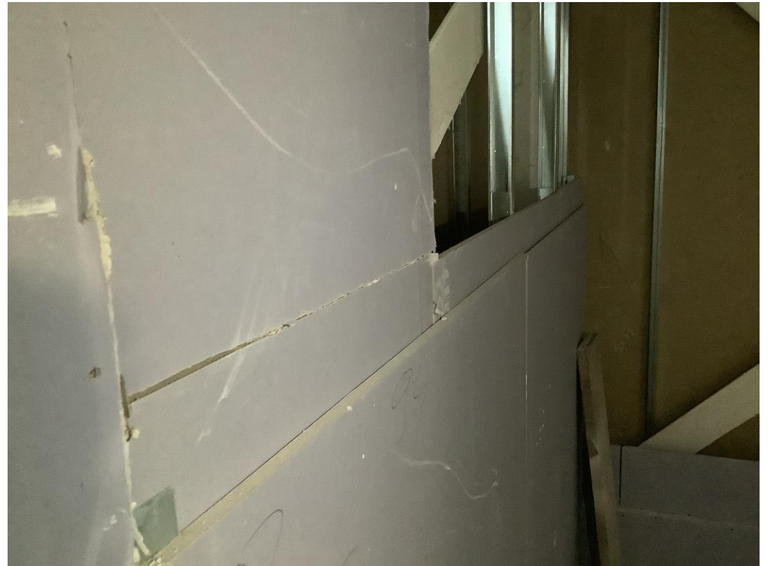
Residential Block – Boarding of metal partitions to circulation areas
