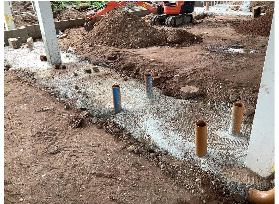
Commercial Block – Under ground drainage
