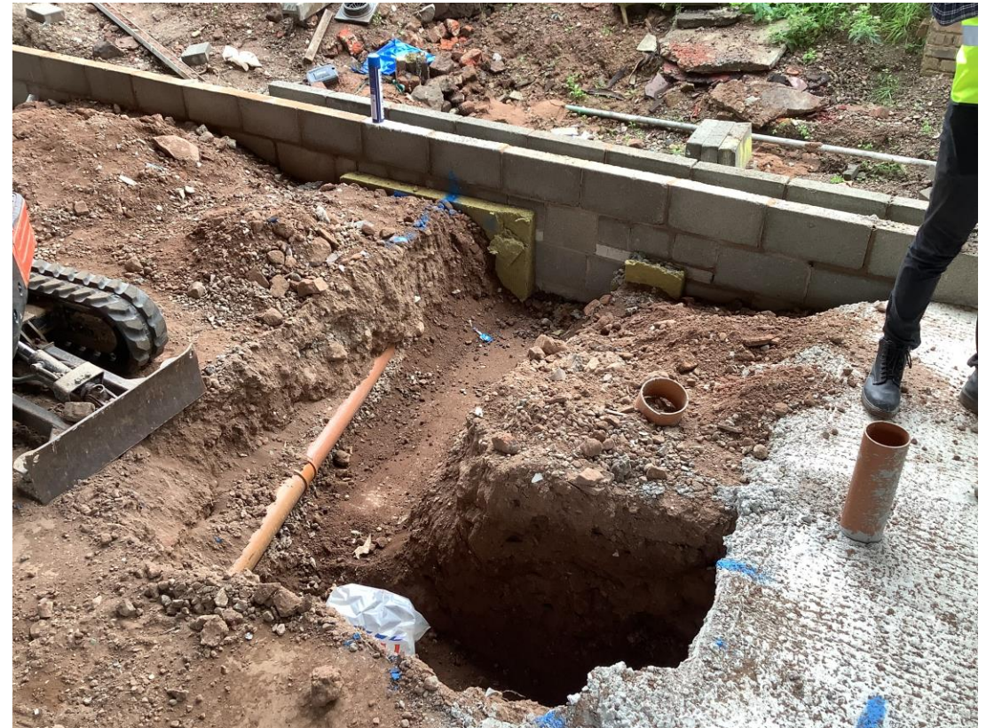
Commercial Block – Under ground drainage
