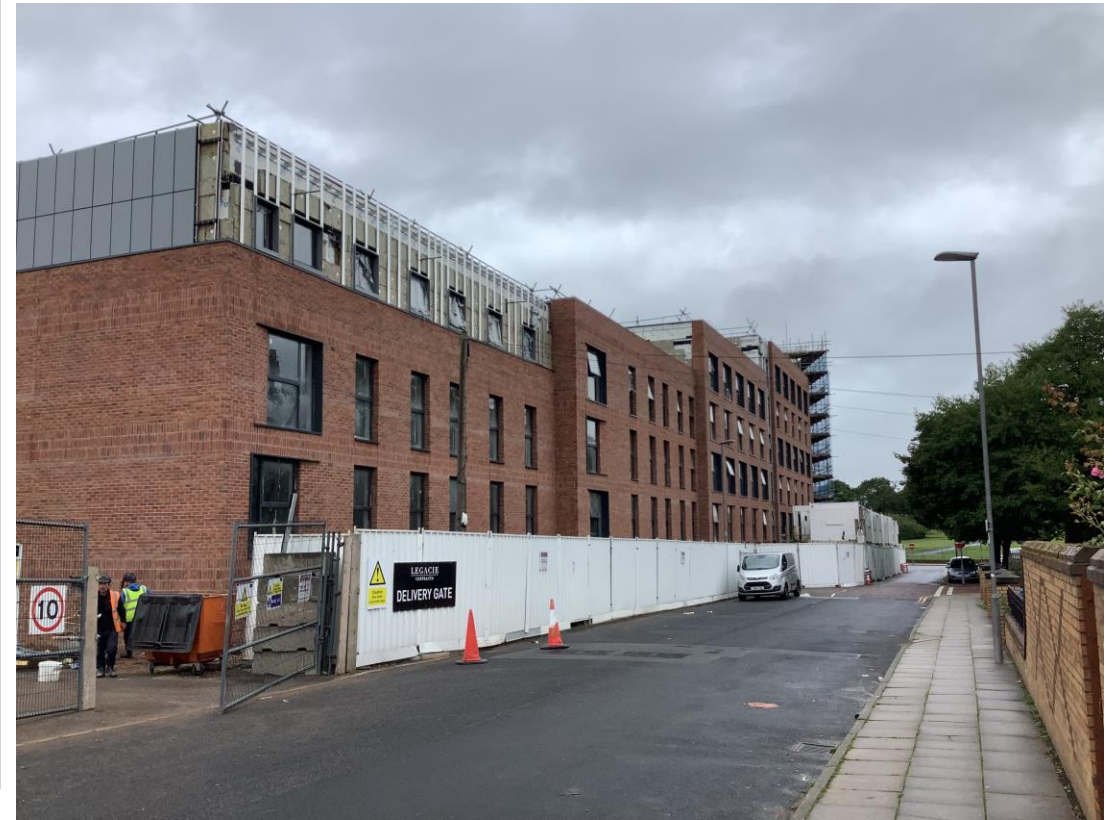
Walker Street - Site view
