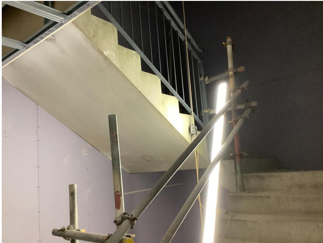
Residential Wing – Handrail & balustrade installation
