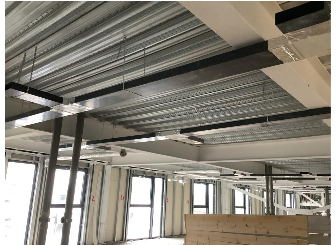
Residential Wing – 1 st Fix Mechanical works
