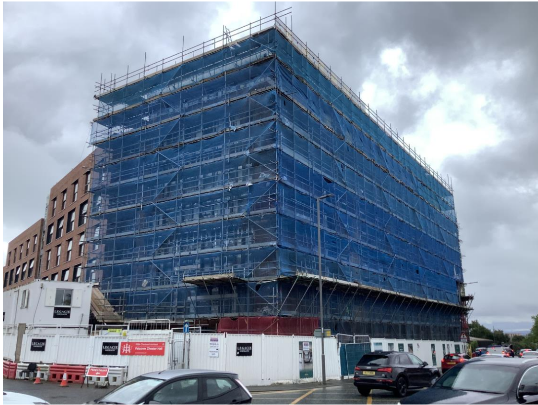
West Derby Road - Site view
