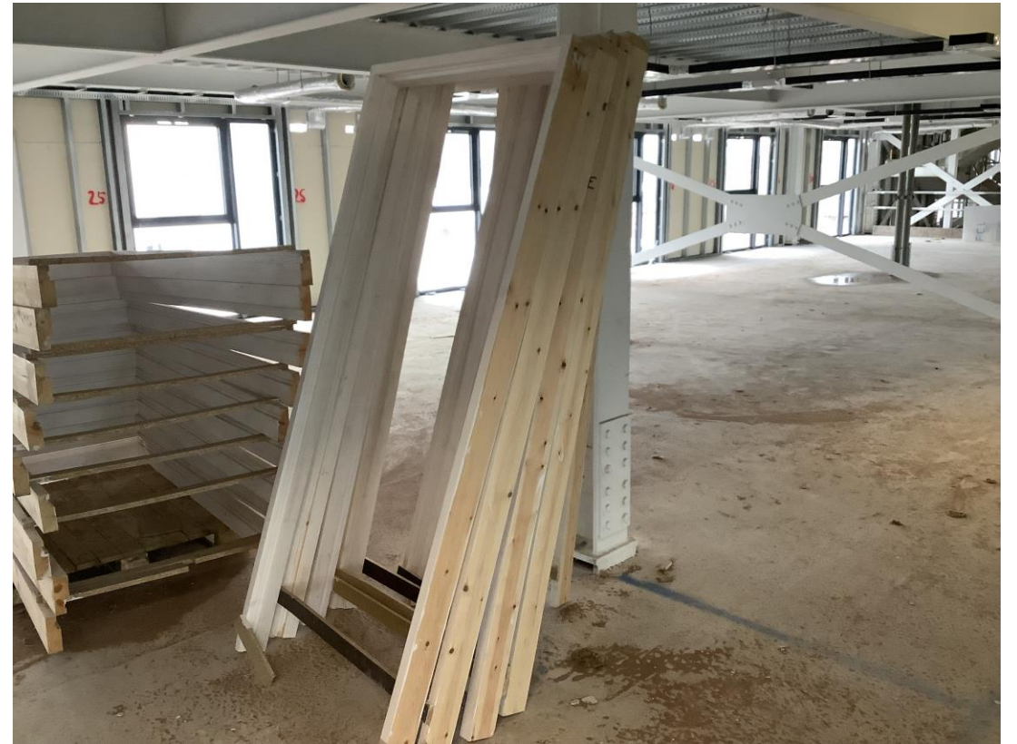
Material storage – Timber door frames
