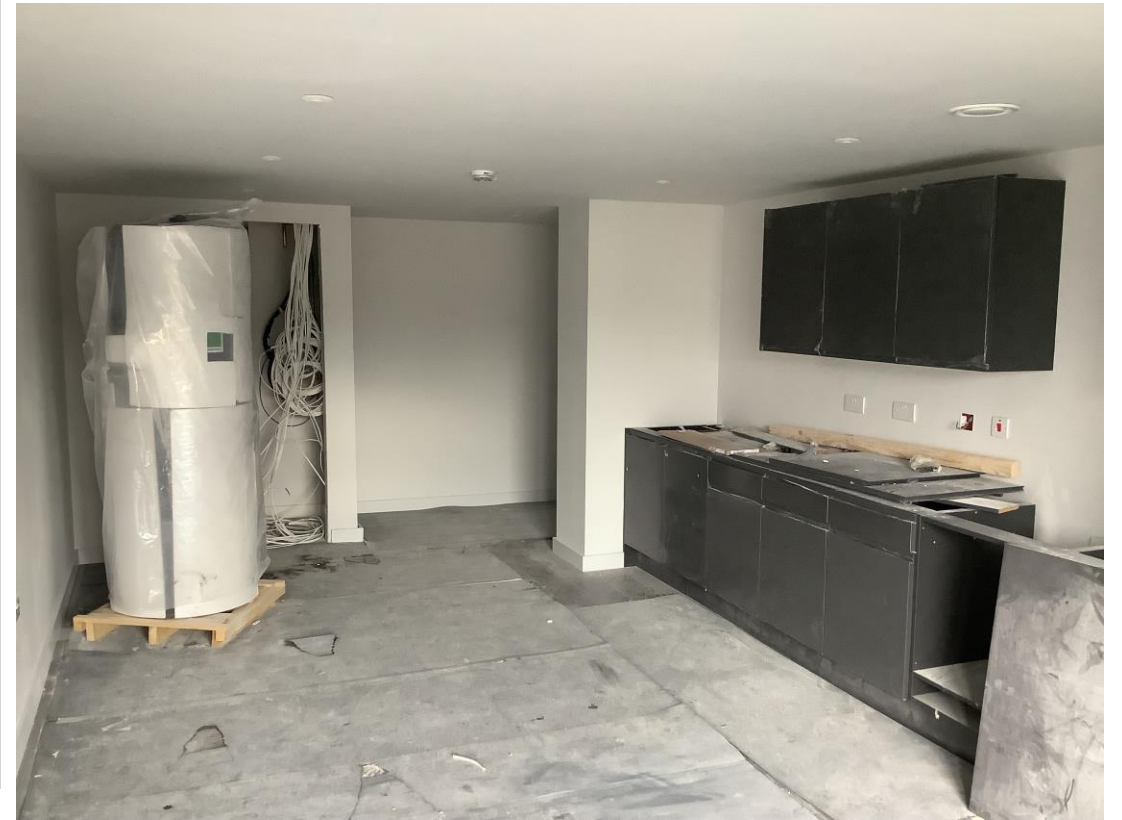
Student Wing – Kitchen units on-going
