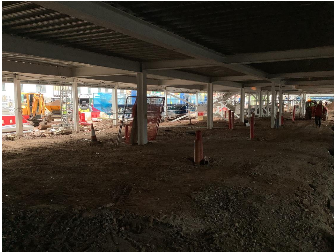
Residential Wing – Under ground drainage works
