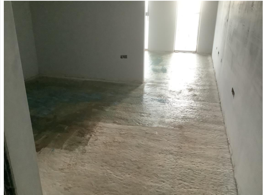
Student Wing – Concrete floor surface preparations
