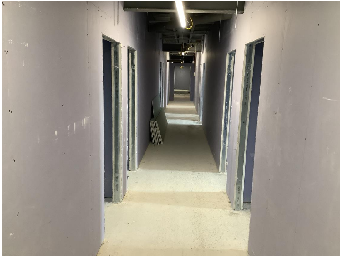
Residential Block – Boarding of partitions to circulation areas
