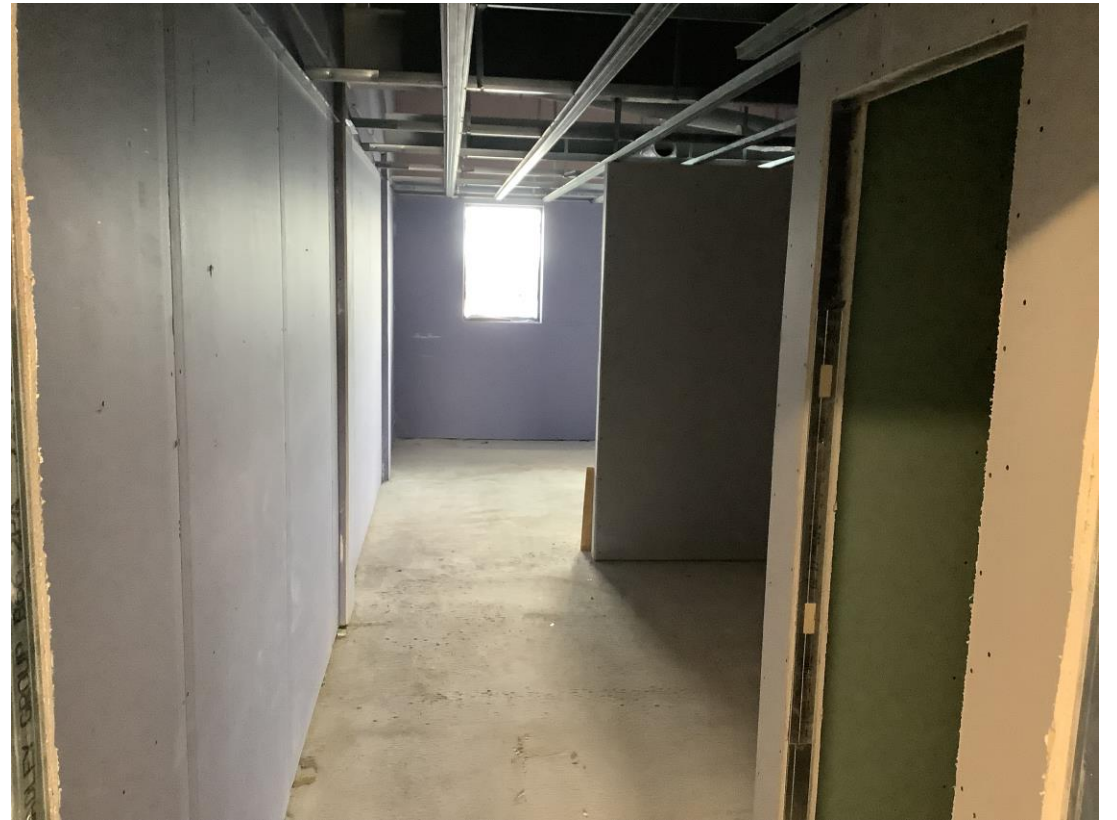
Residential Block – Boarding of partitions & erection of metal ceiling
