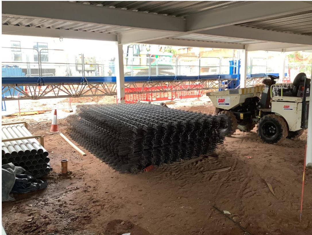
Material storage – Steel reinforcement
