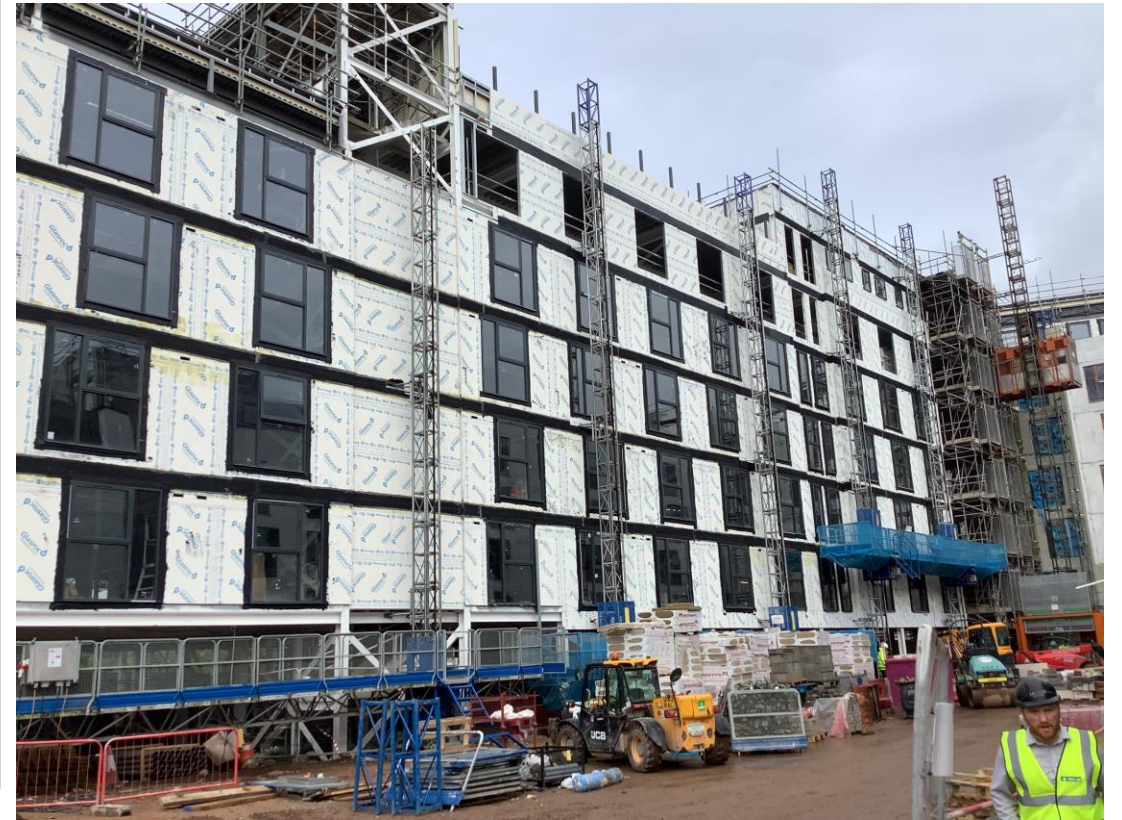
Residential Wing – Mast climbers installed to inner courtyard elevation
