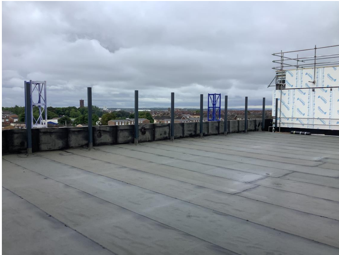
Commercial Block – External metal balustrade
