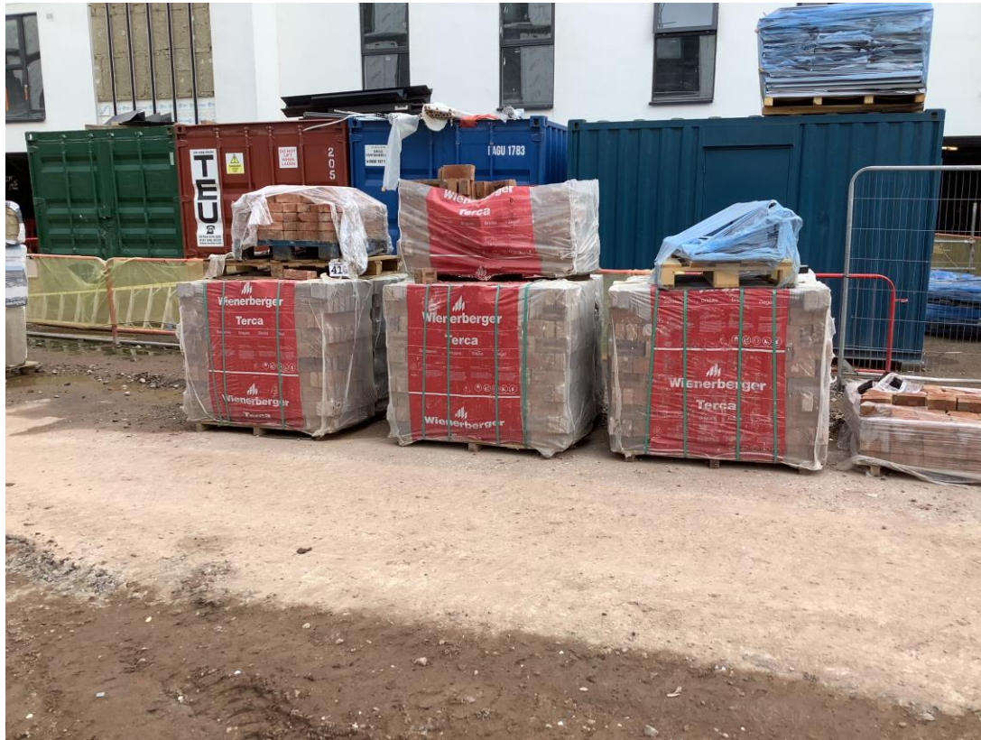
Material storage – Red brick
