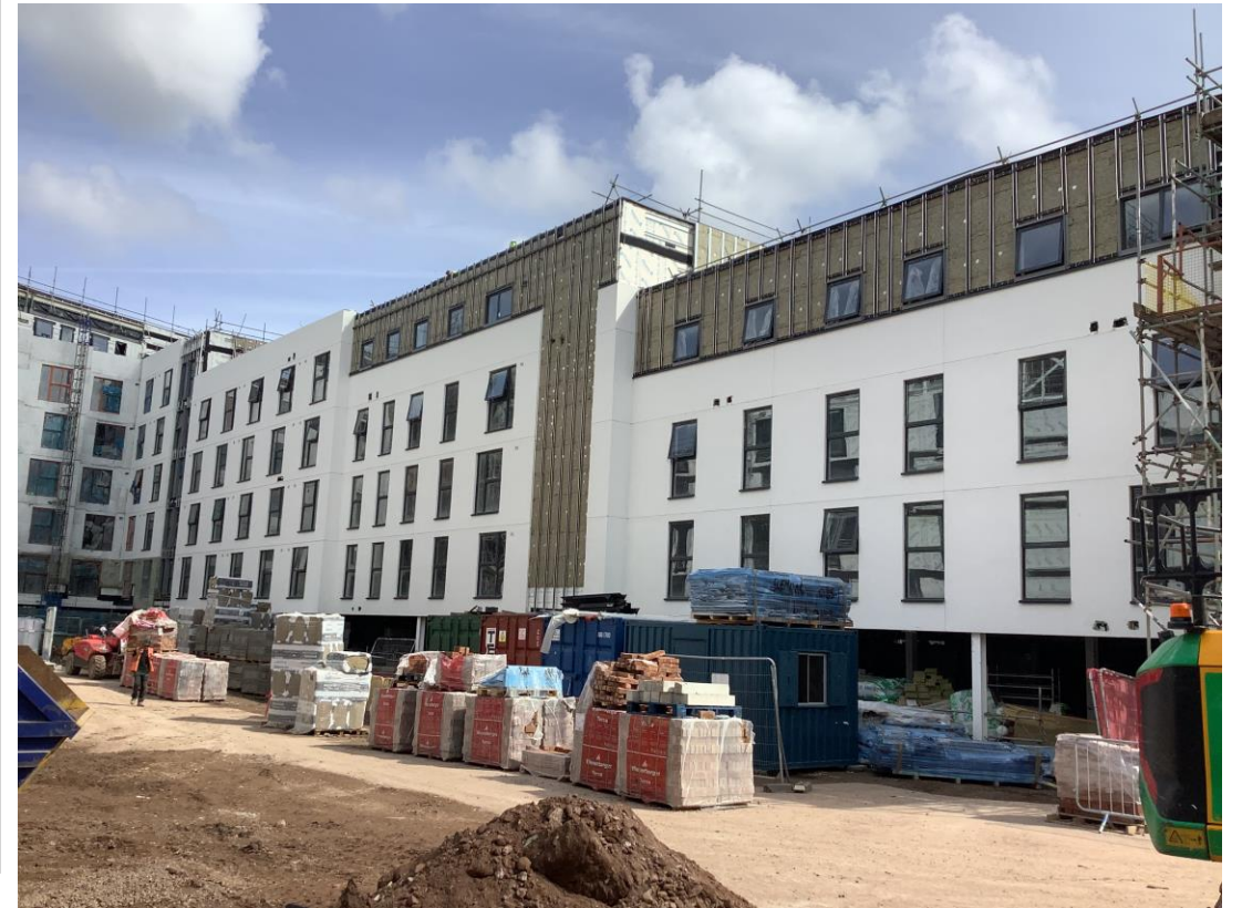
Student Wing – Render application & cladding progress
