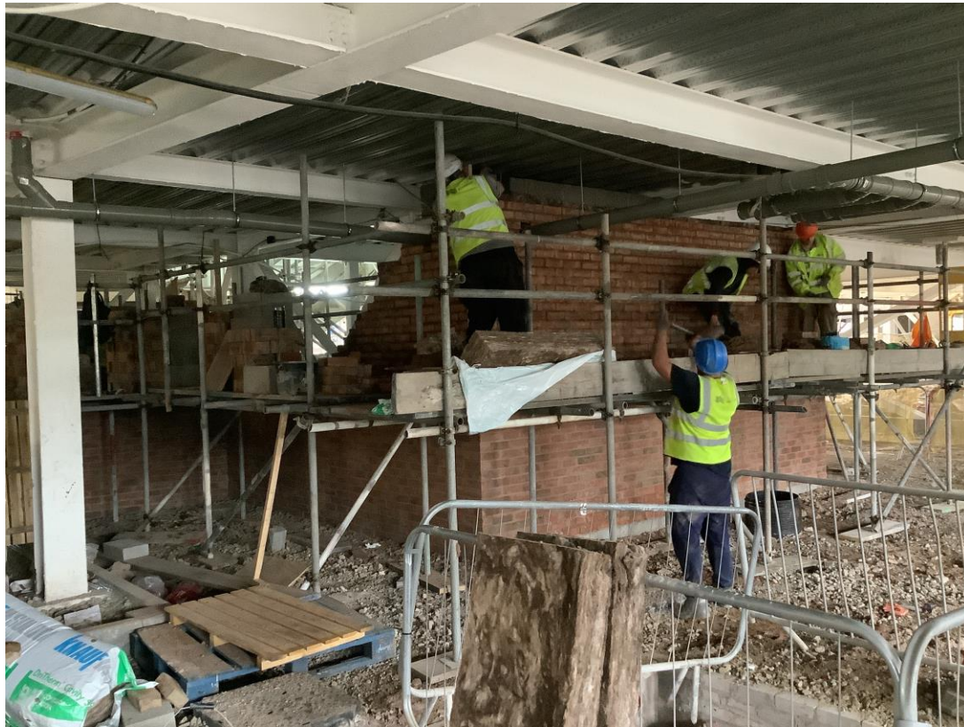
Brickwork to stair core on-going
