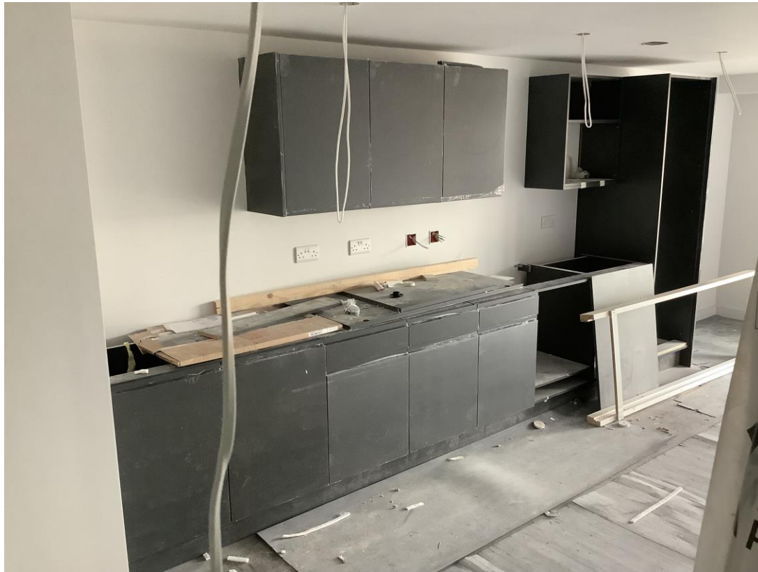
Student wing – Kitchen units on-going
