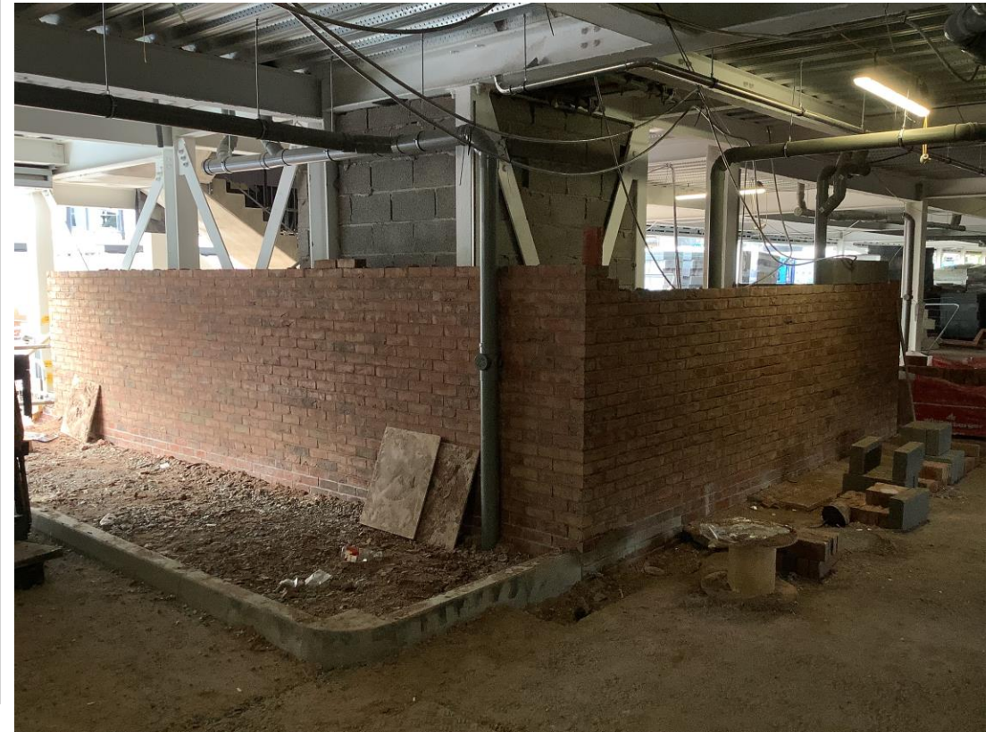
Brickwork to stair core
