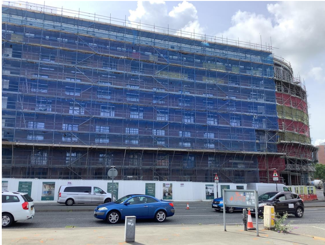
West Derby Road - Site view
