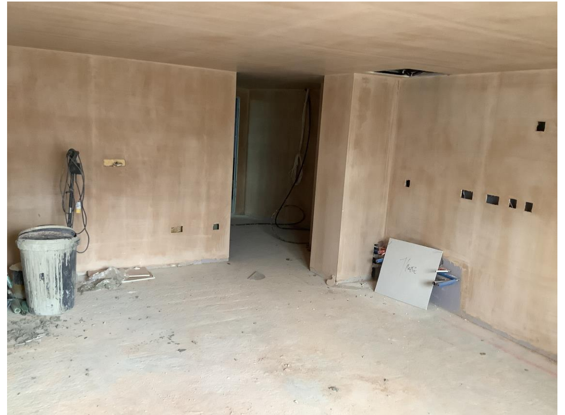
Residential wing – Plastering to internal walls
