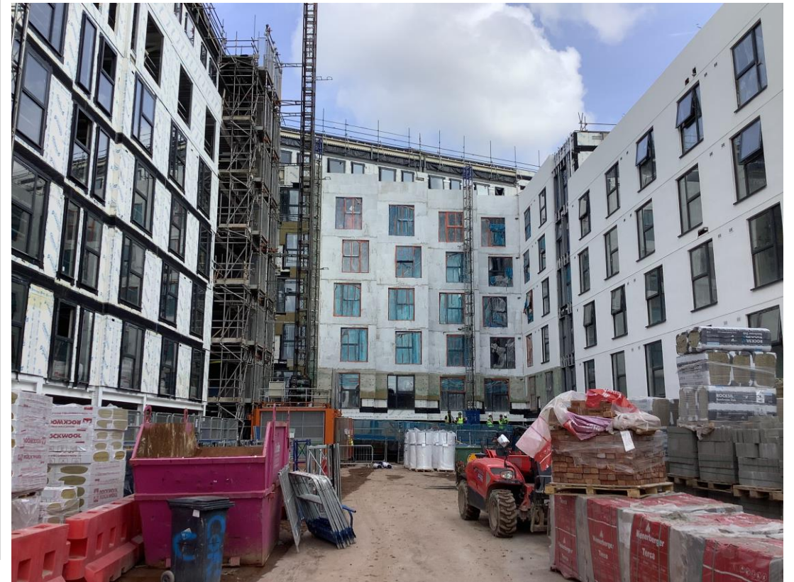
'Zig-zag' elevation - General progress photo
