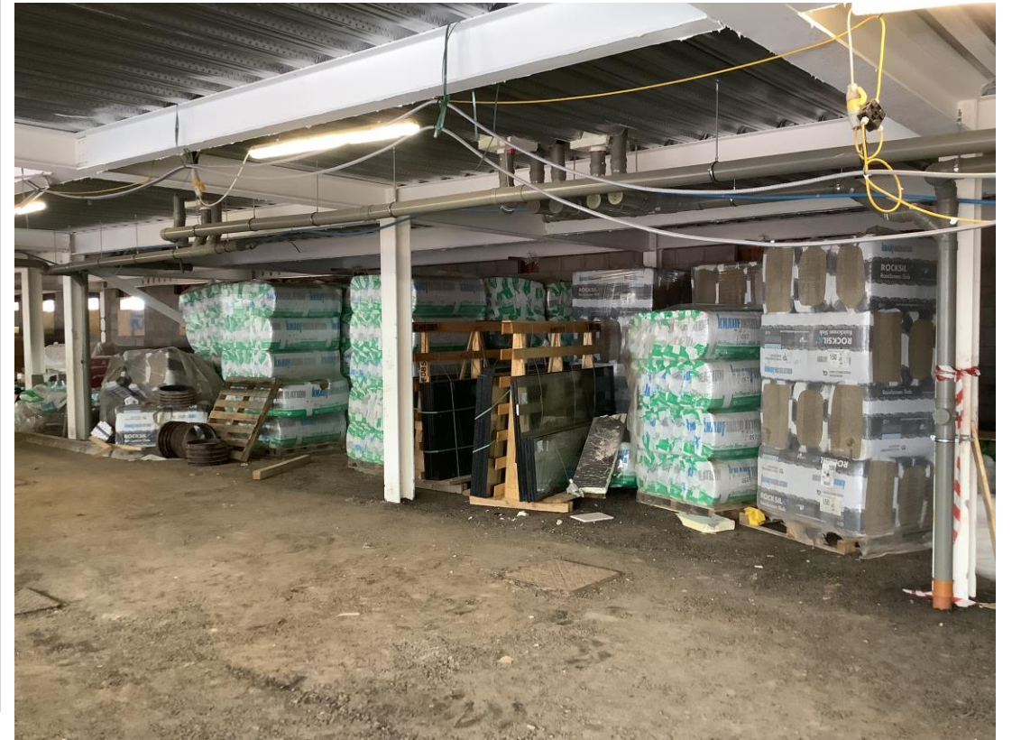
Material storage – Insulation and glazing panels
