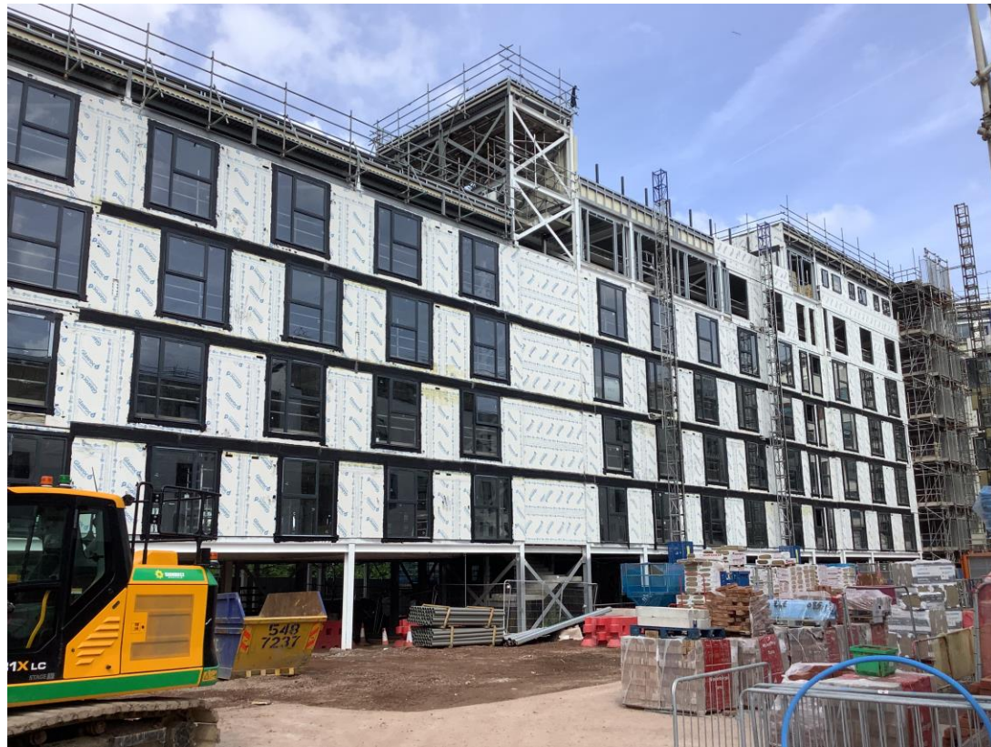
Residential Wing – Render application & cladding progress
