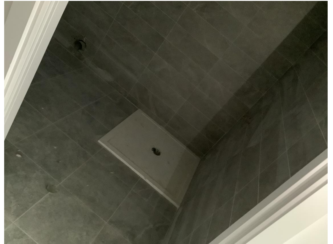
Student wing – DDA bathroom fitting on-going
