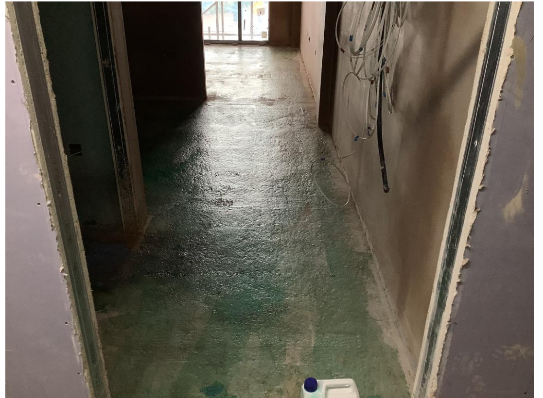
Residential wing – Self levelling screed preparation
