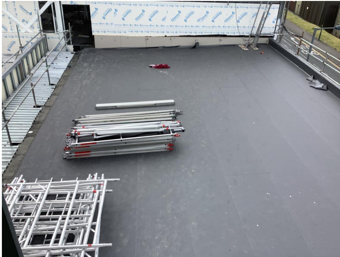
Commercial block – Flat roof coverings progress
