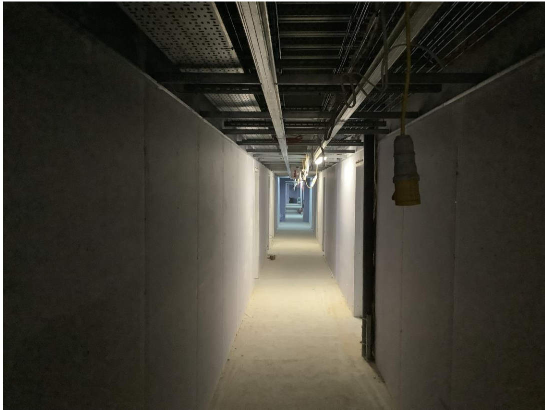
Residential wing – Boarding of partitions on-going
