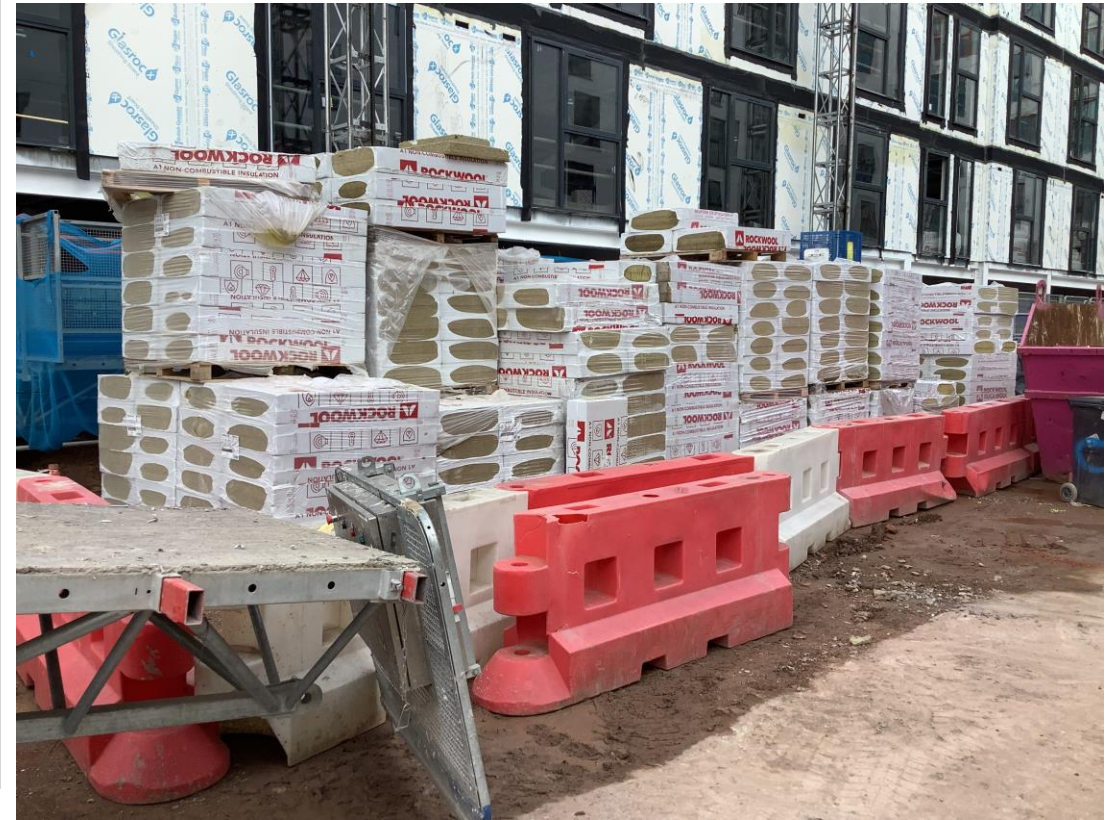
Material storage – Rockwool insulation
