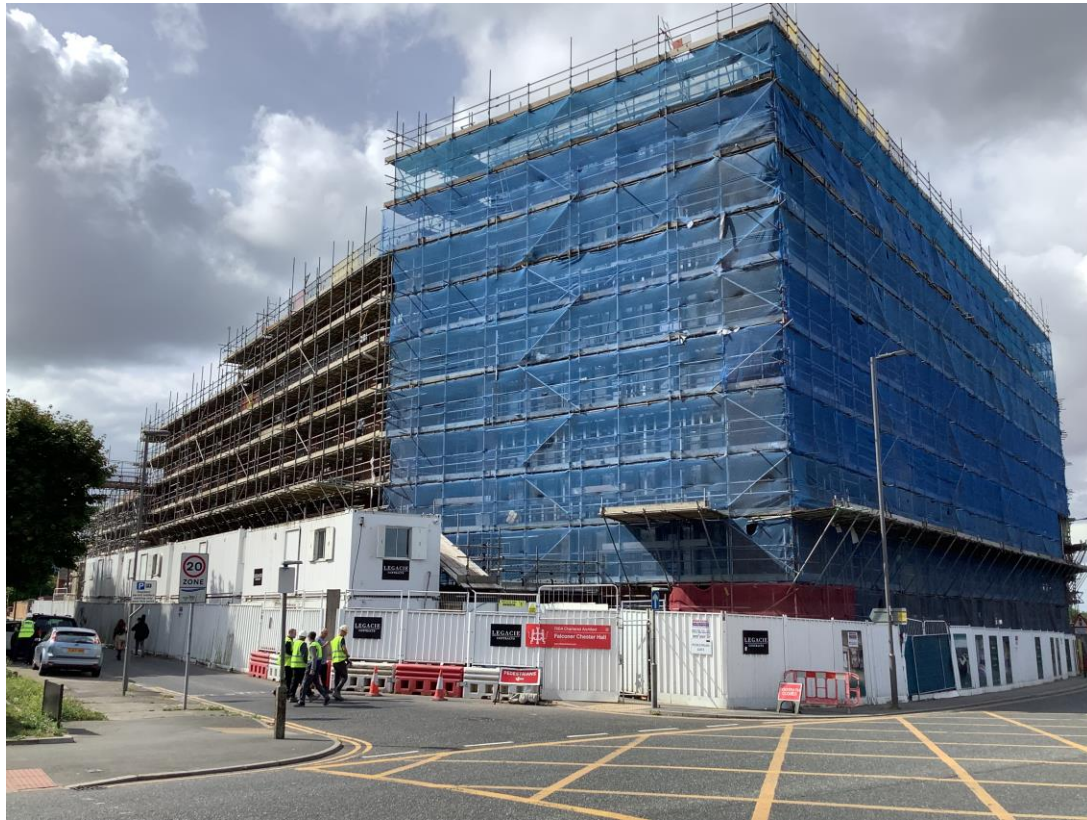
West Derby Road - Site view
