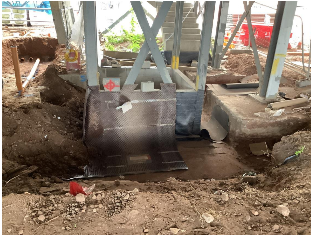
Lift core tanking
