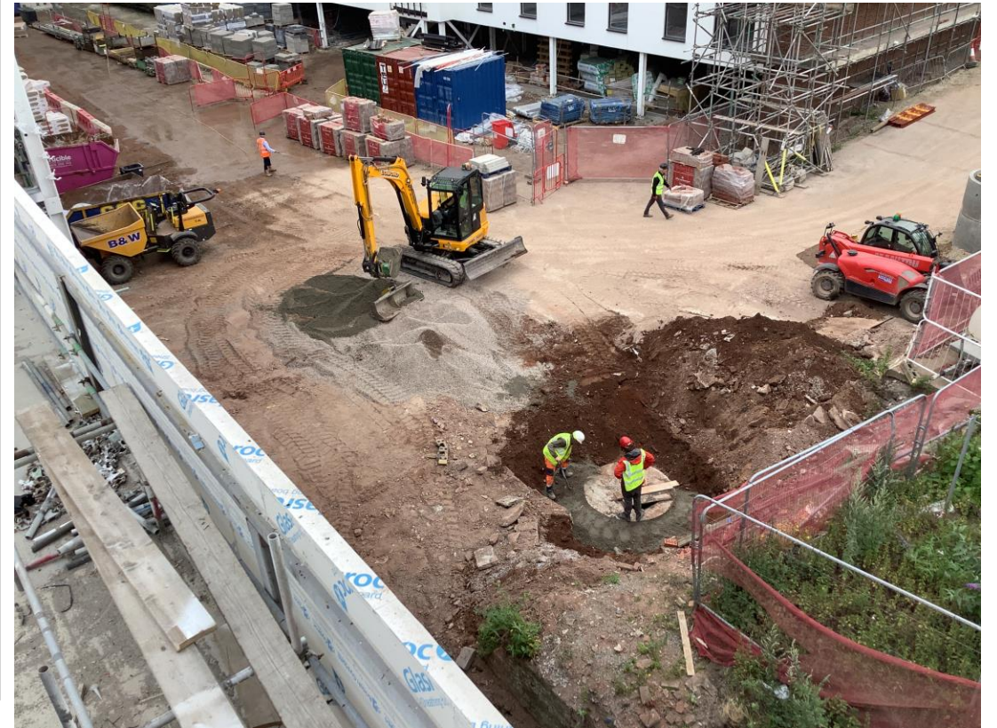
External excavation works
