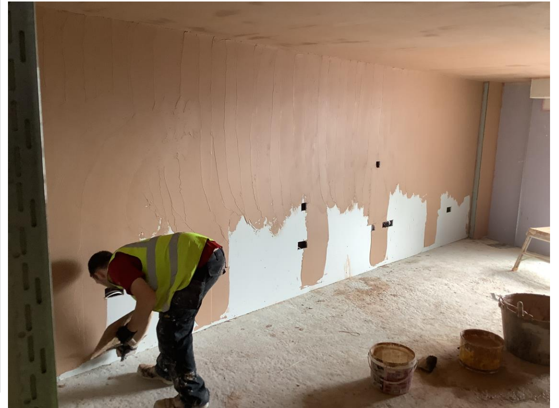
Residential wing – Plastering to internal walls on-going
