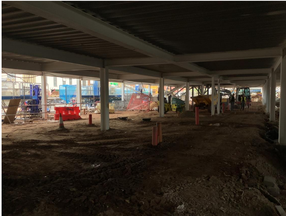
Ground Floor drainage works
