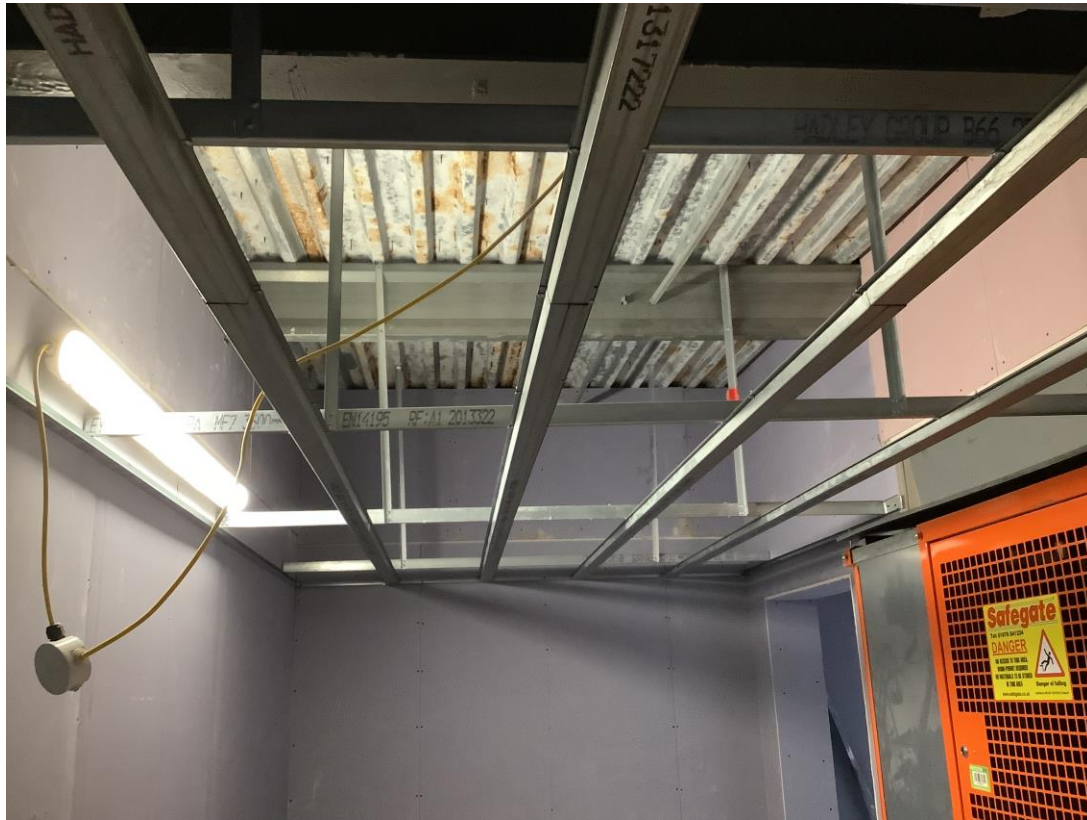
Student wing / Upper floors – Metal frame ceiling
