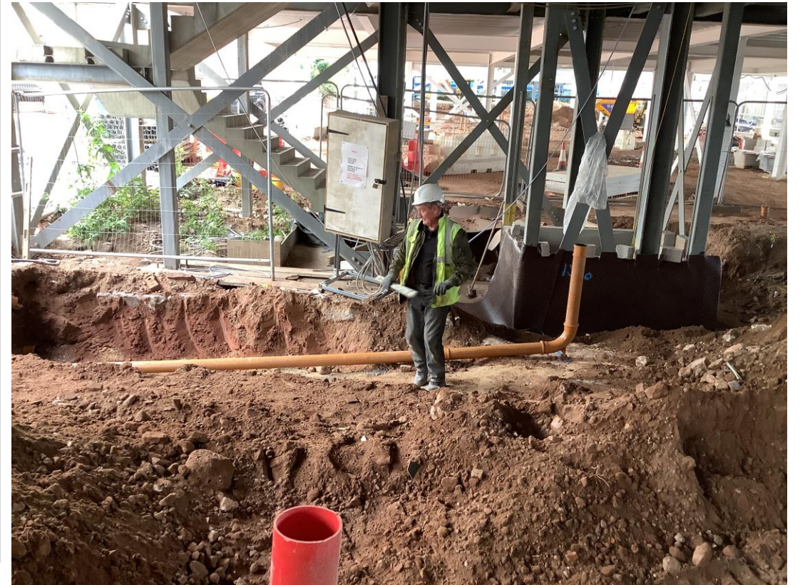
Ground Floor drainage works
