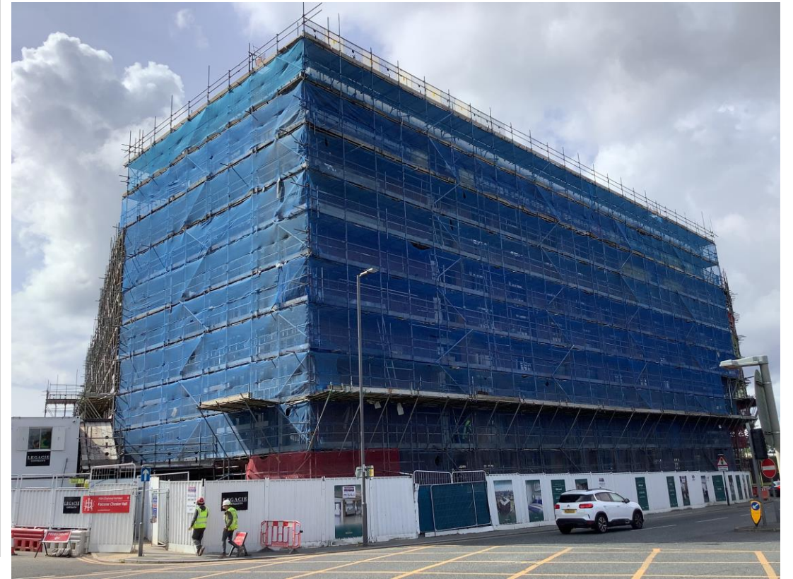
West Derby Road - Site view
