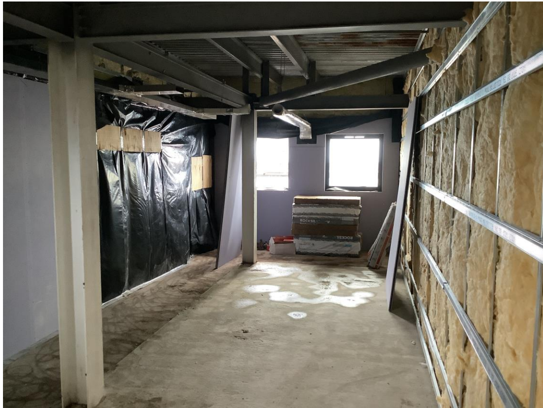
Student wing / Upper floors – Insulation & boarding of partition walls
