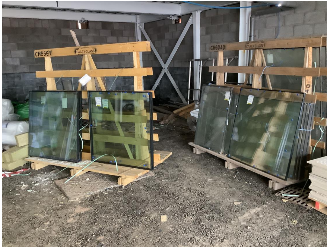
Material storage – Glazing panels
