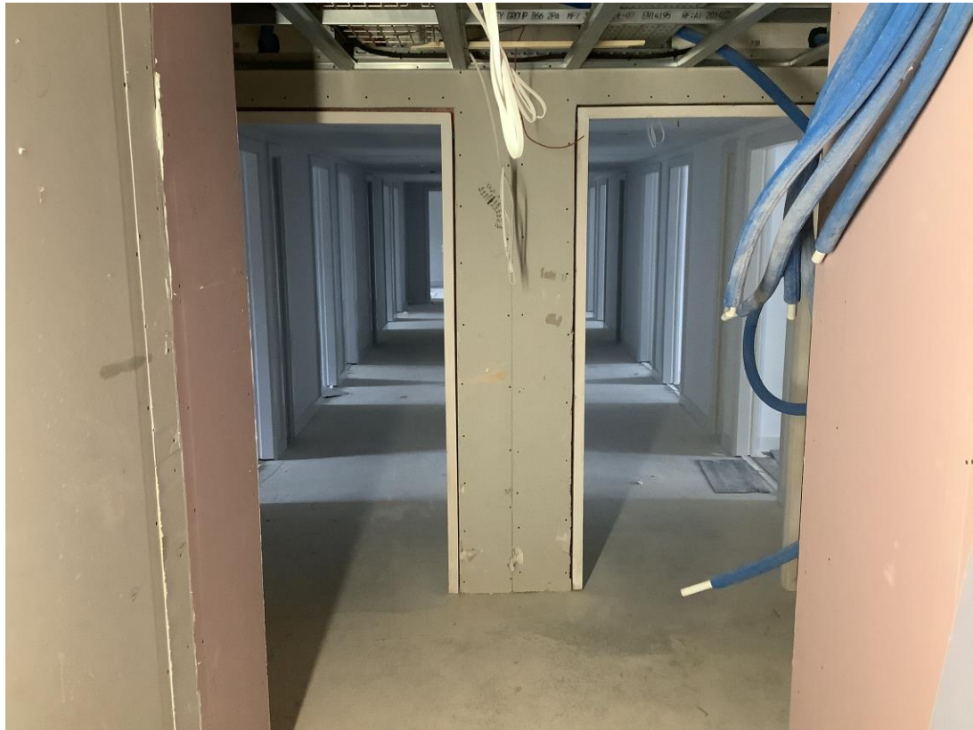
Student wing – Plasterboard & joinery
