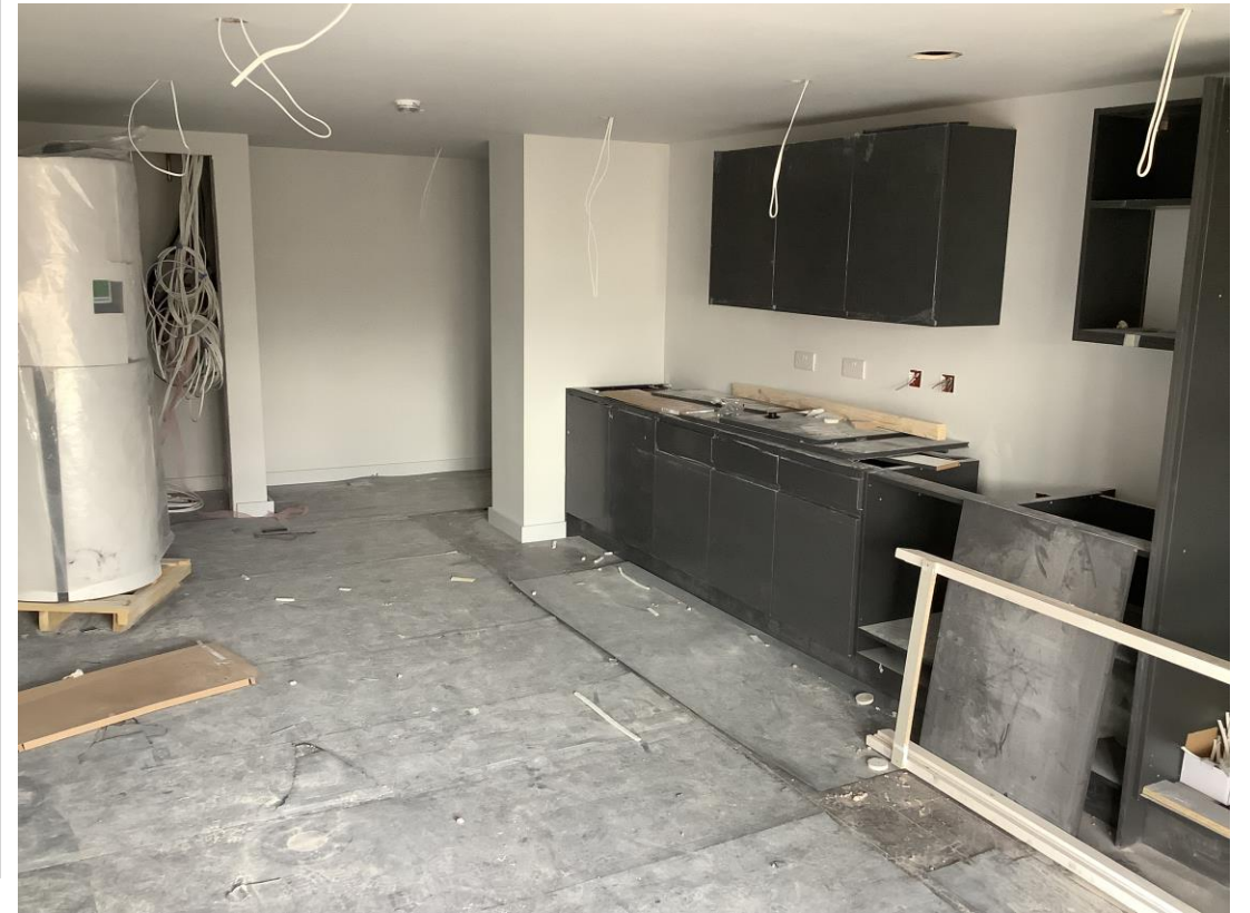
Student wing – Kitchen units on-going
