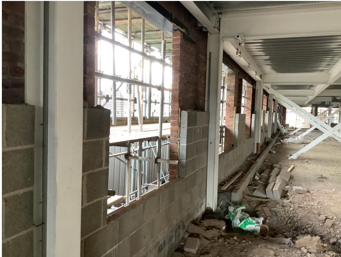
External wall brick & blockwork
