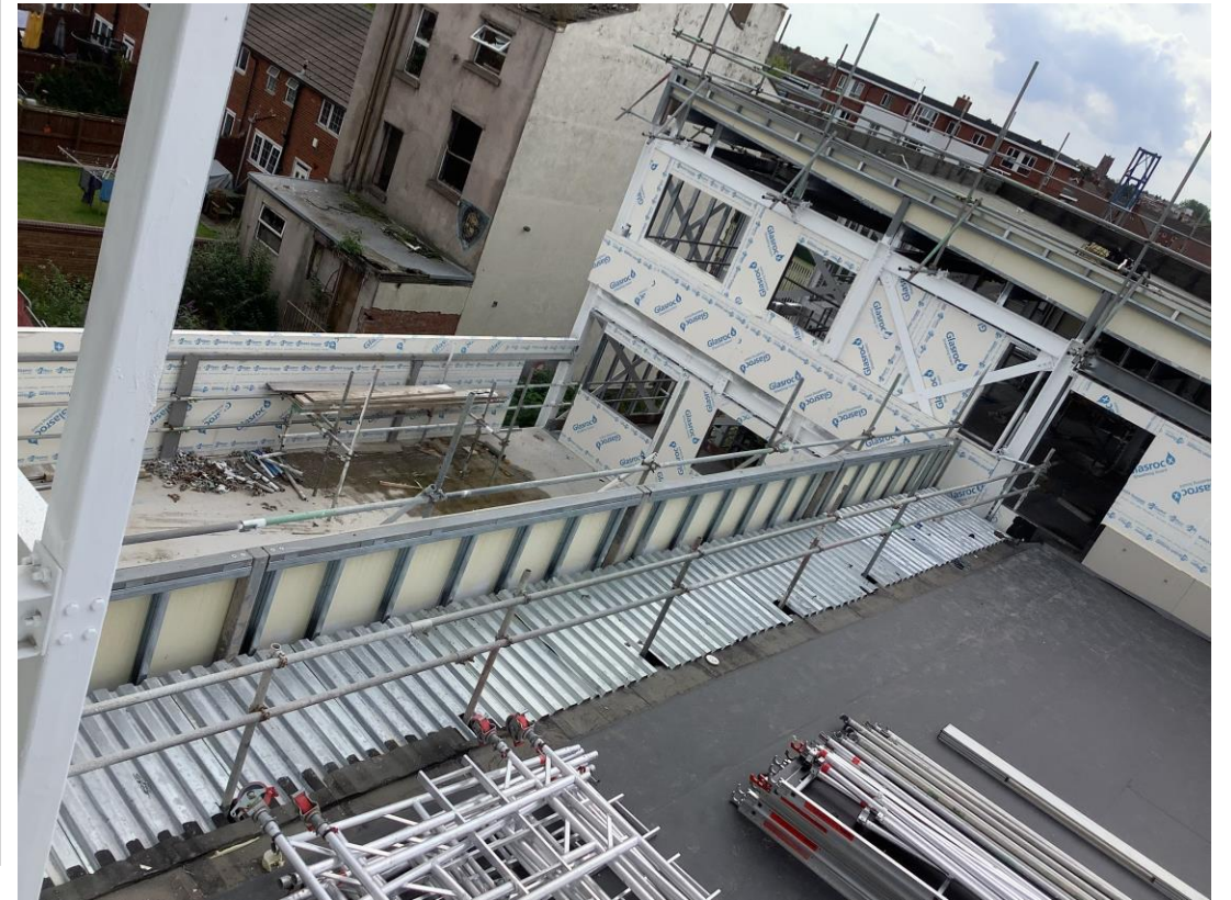
Commercial block – SFS & weatherboarding
