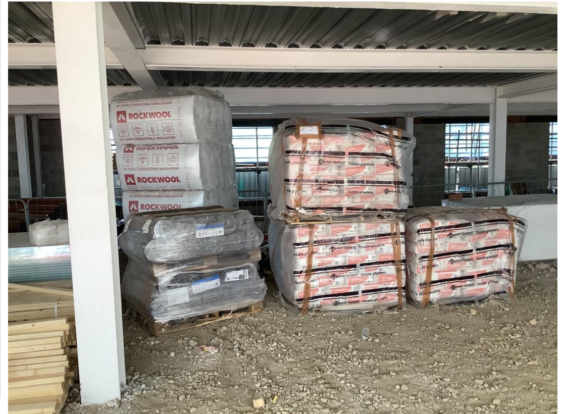
Material storage – Gypsum plaster
