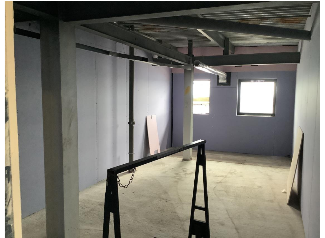
Student wing / Upper floors – Boarding of partition walls
