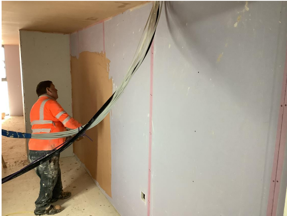
Residential wing – Plastering to internal walls on-going
