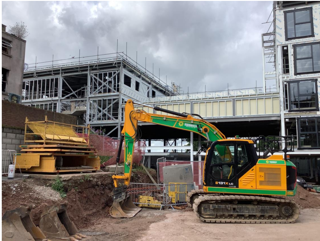
Commercial Block - SFS, weatherboard and windows
