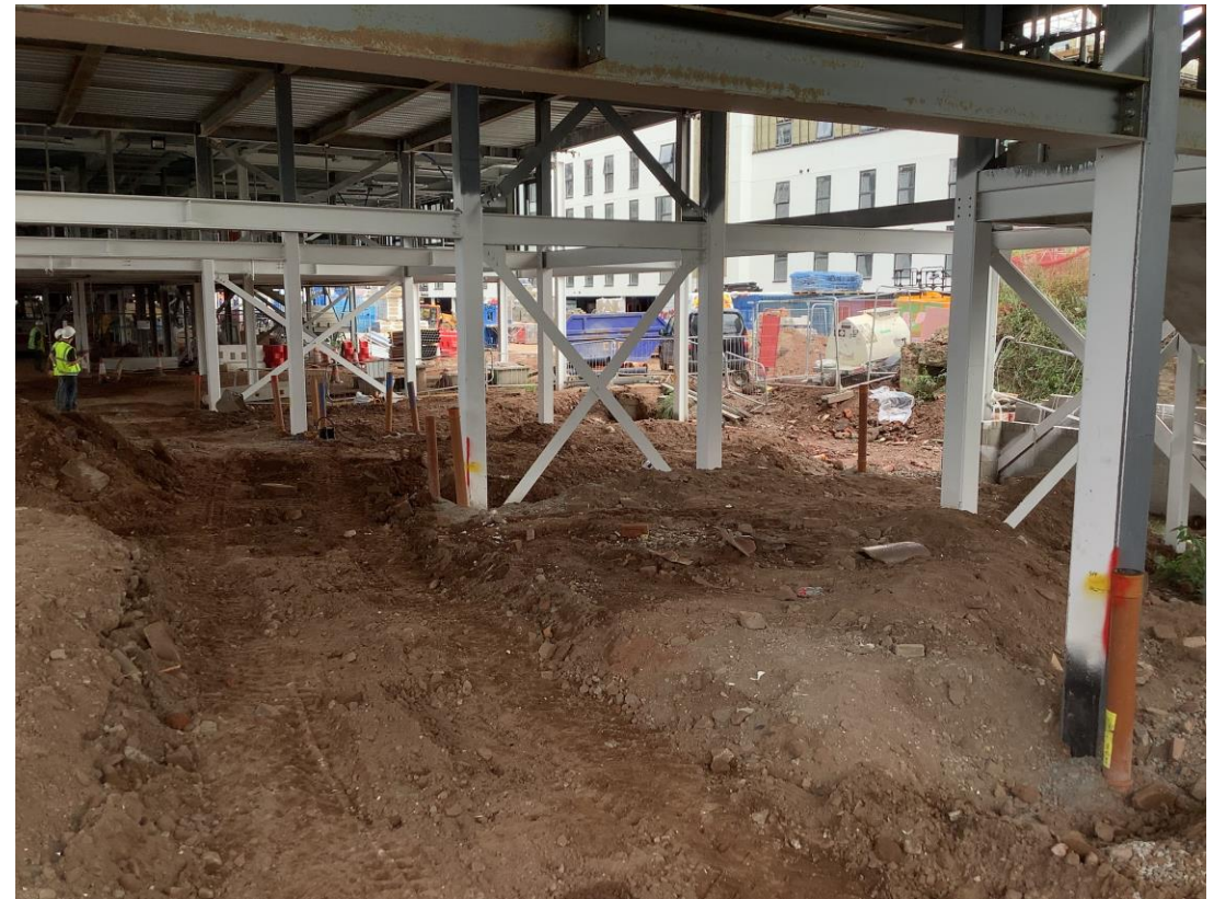
Ground Floor drainage works
