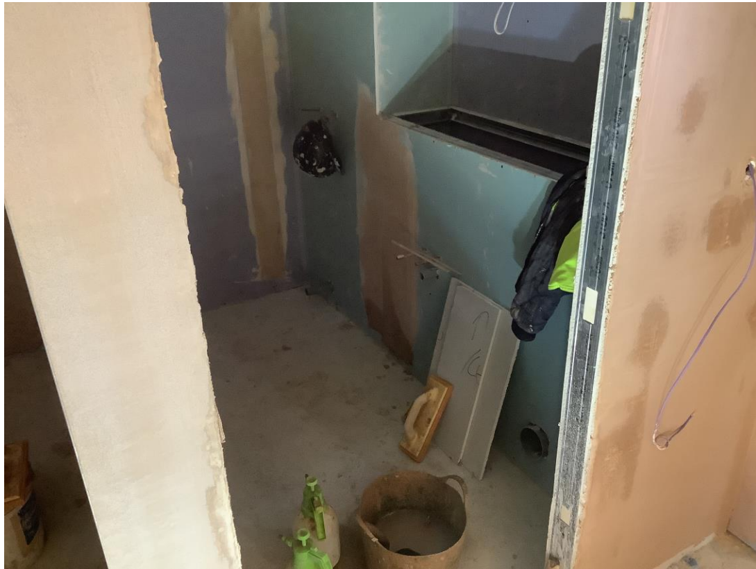
Residential wing – Boarding of recessed drainage installation
