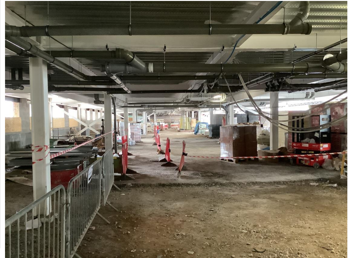
Student wing – Undercroft parking progress
