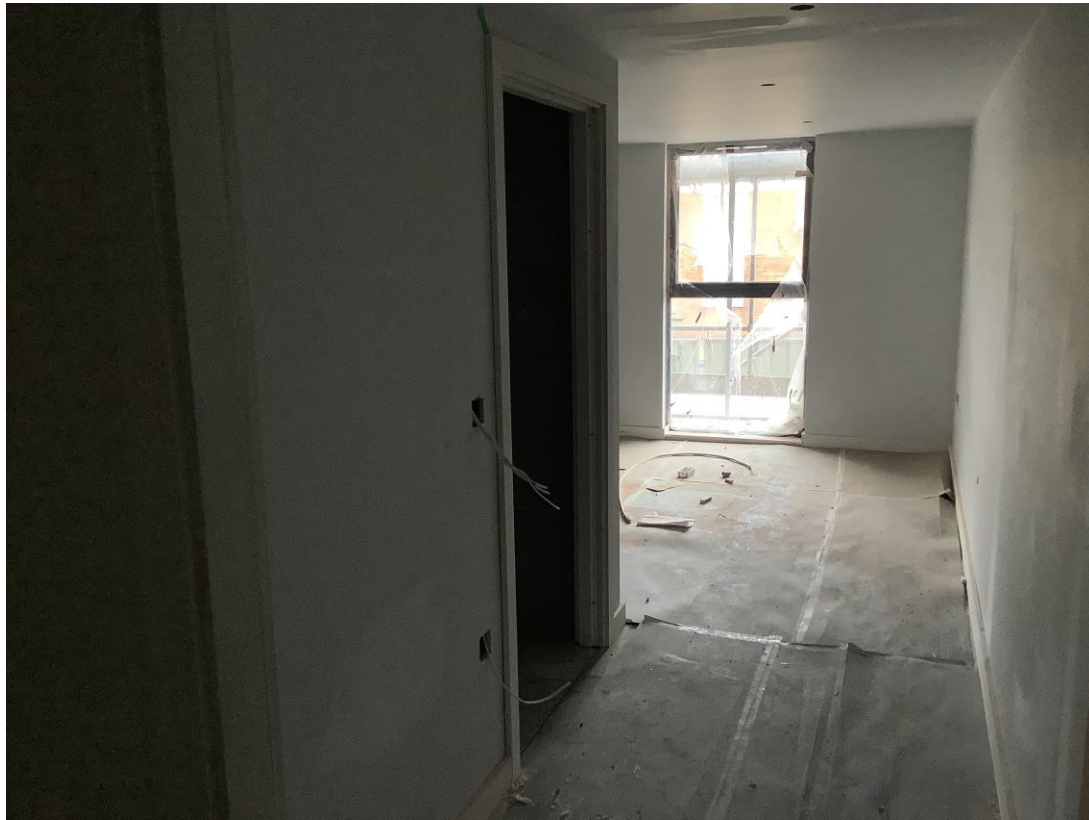
Student wing – Joinery, floor finishes and internal decorations
