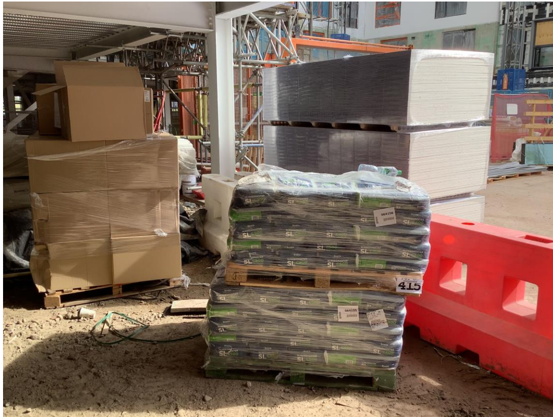
Material storage – Self-levelling screed
