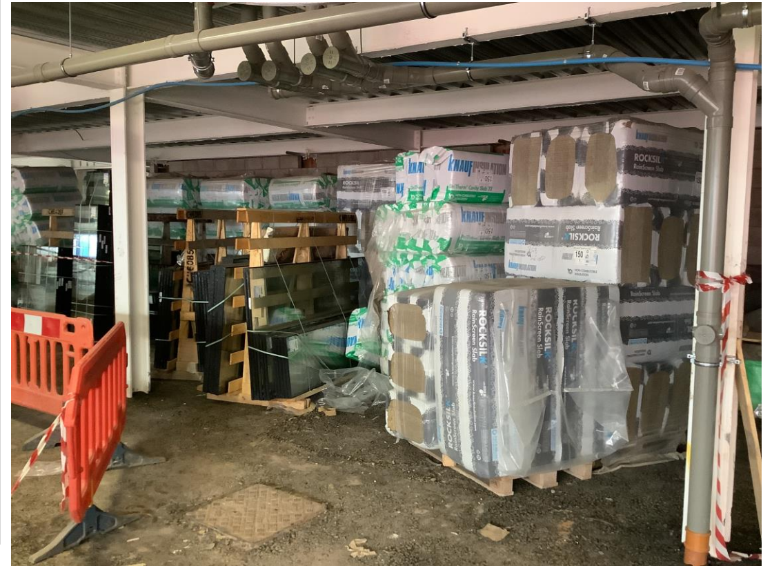
Material storage – Insulation and glazing panels
