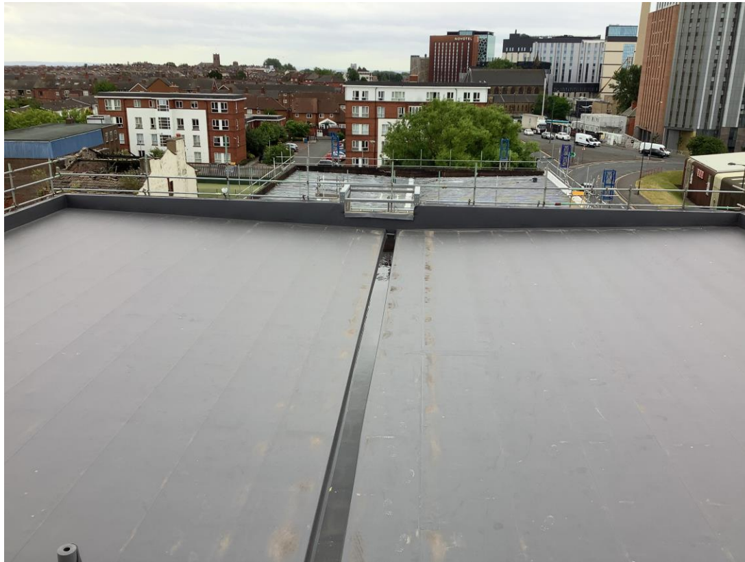
Residential wing – Flat roof coverings progress
