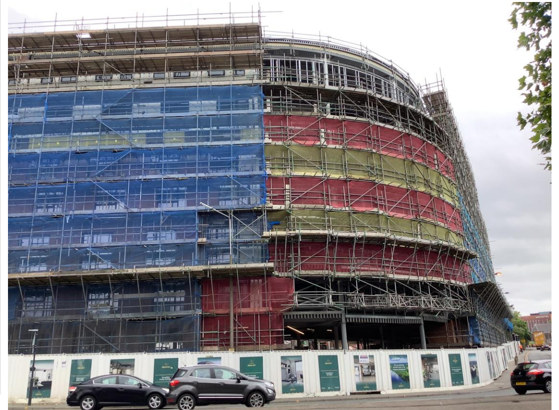
West Derby Road - Site view
