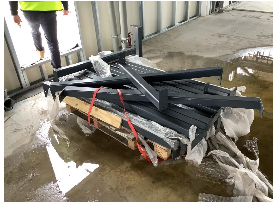
Material storage – Cross sections to external ballustrade
