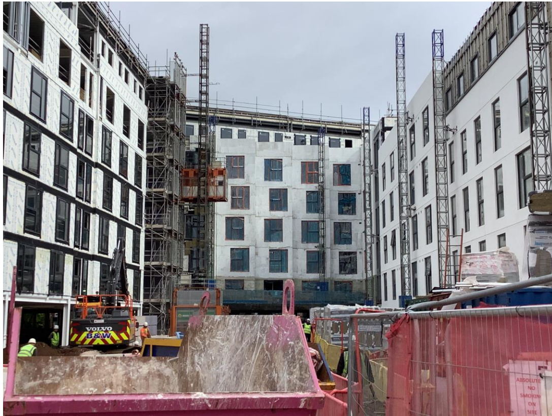
'Zig-zag' elevation - General progress photo
