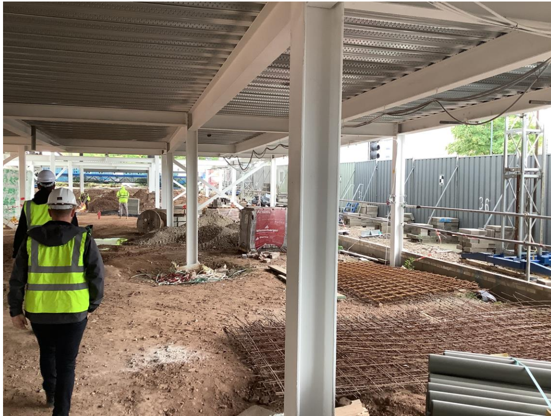
Residential wing – Fire coating steelwork
