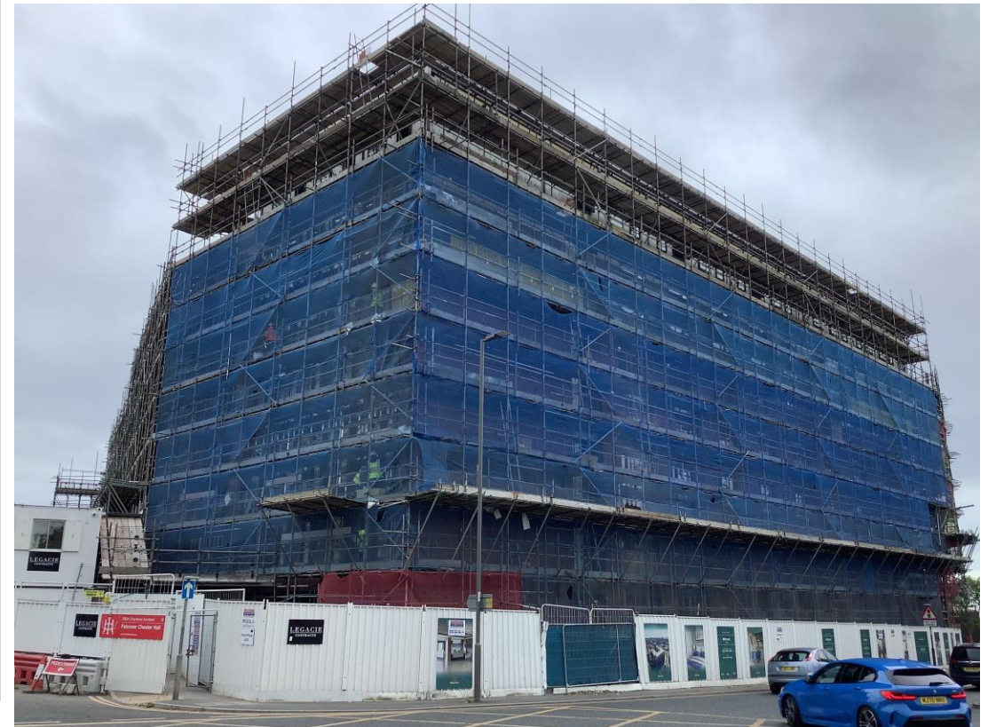
West Derby Road - Site view
