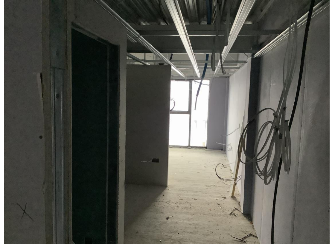
Residential wing – Boarding of partitions on-going
