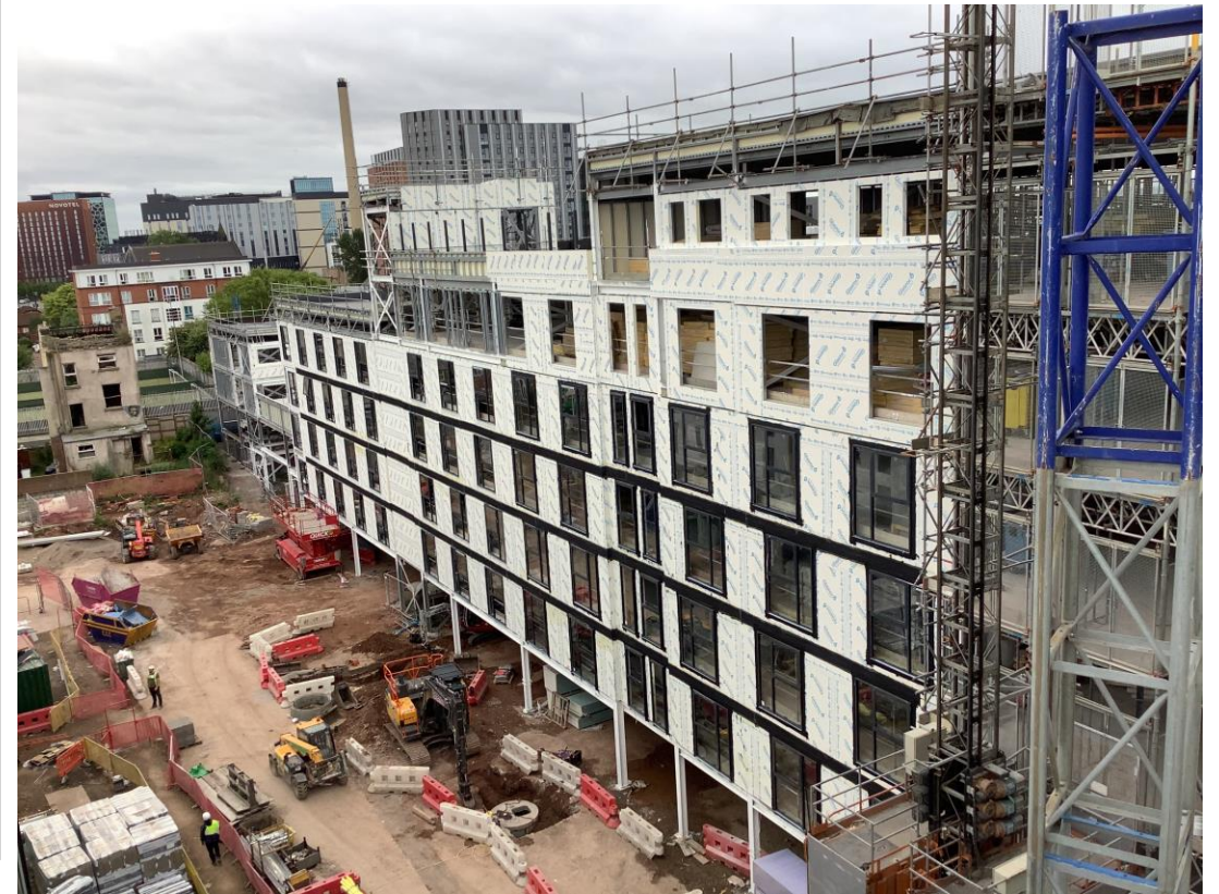
Residential wing – SFS, weatherboard and windows
