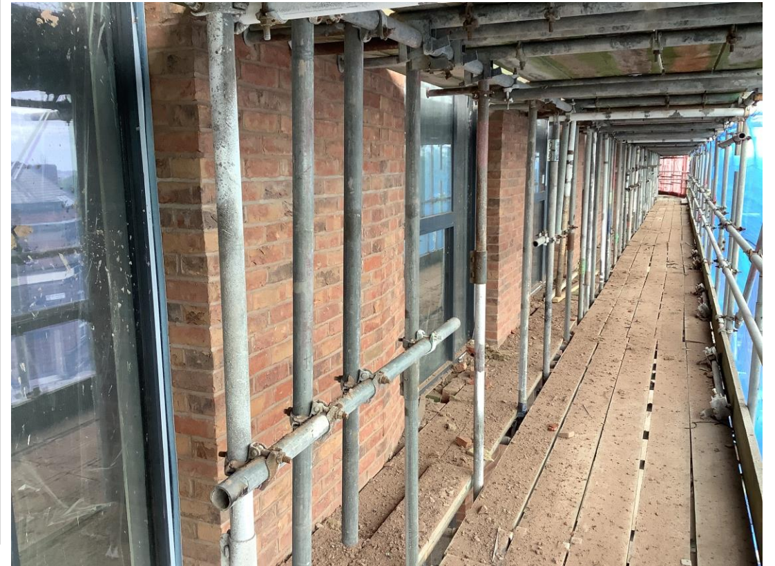
Residential wing – External brickwork on-going
