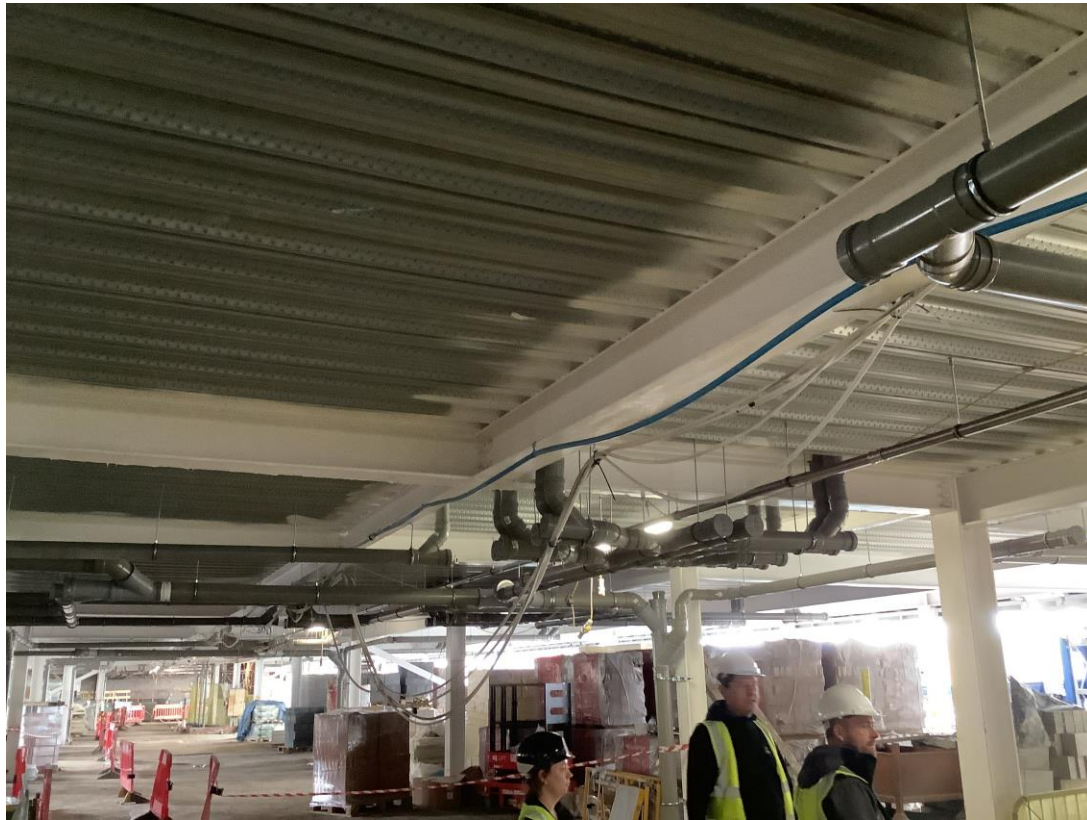
Student wing – 1 st fix M&E on-going
