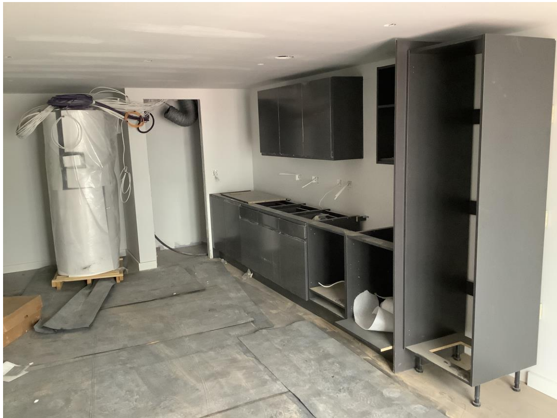
Student wing – Kitchen units on-going
