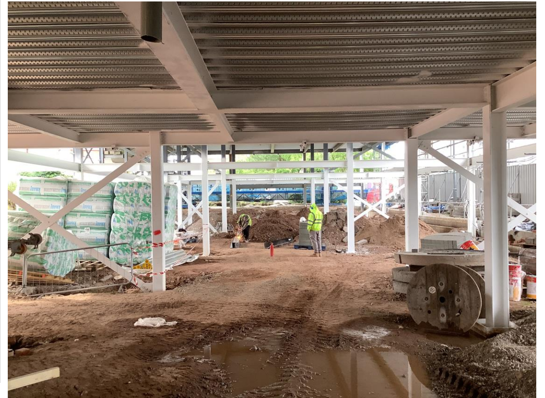
Commercial block – Fire coating steelwork
