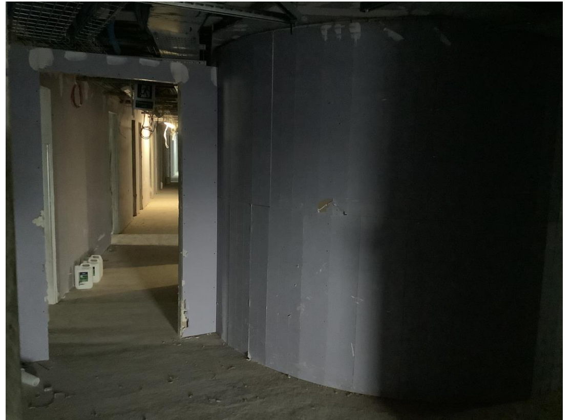
Student wing – Boarding of partitions on-going
