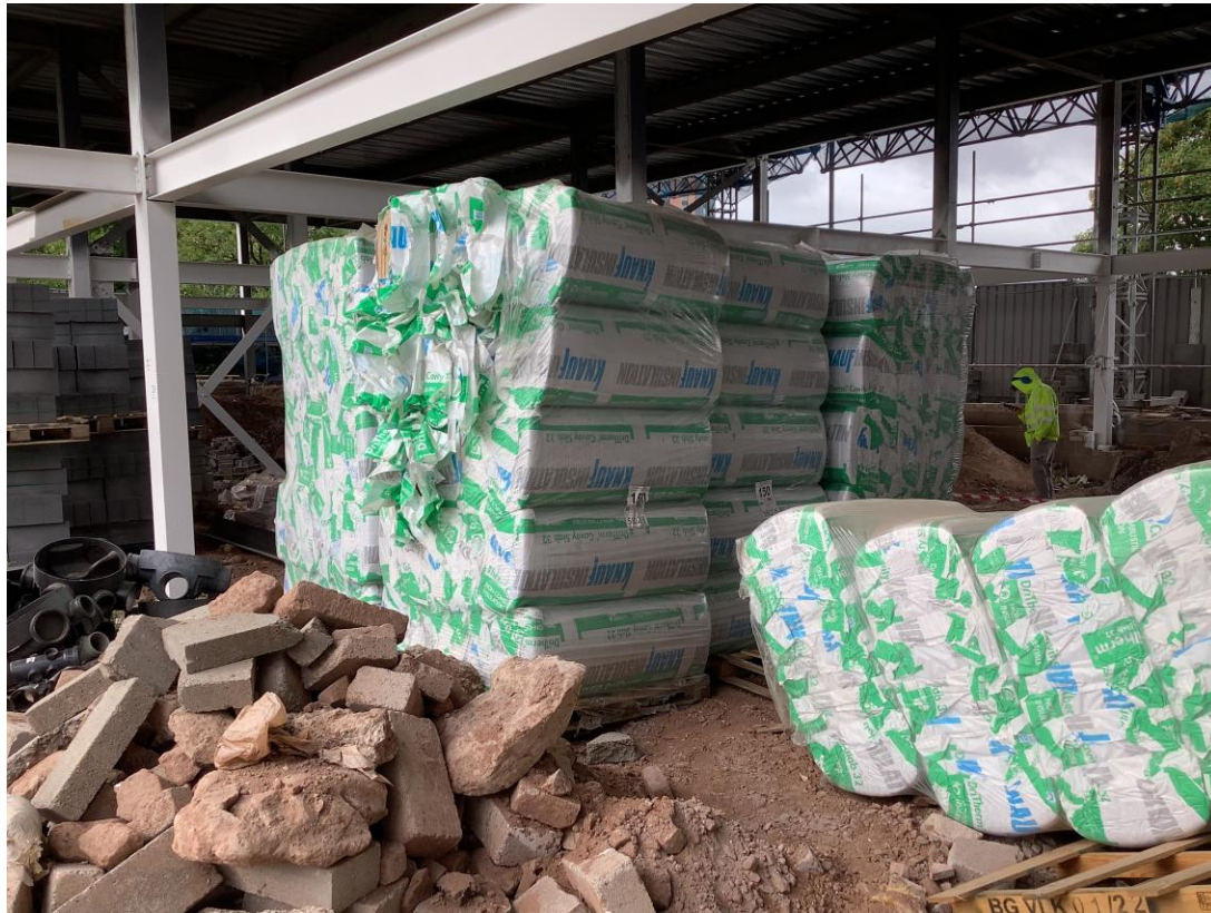
Material storage – Knauf insulation
