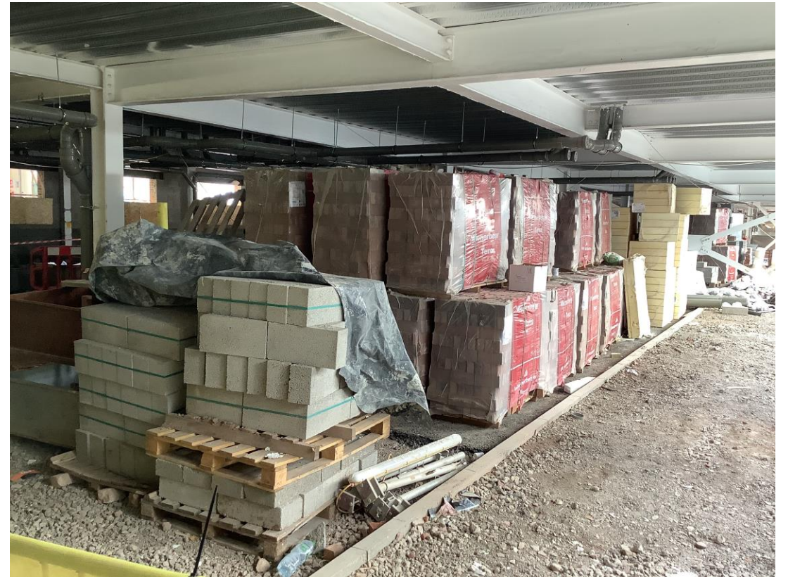
Material storage – Block and red brick
