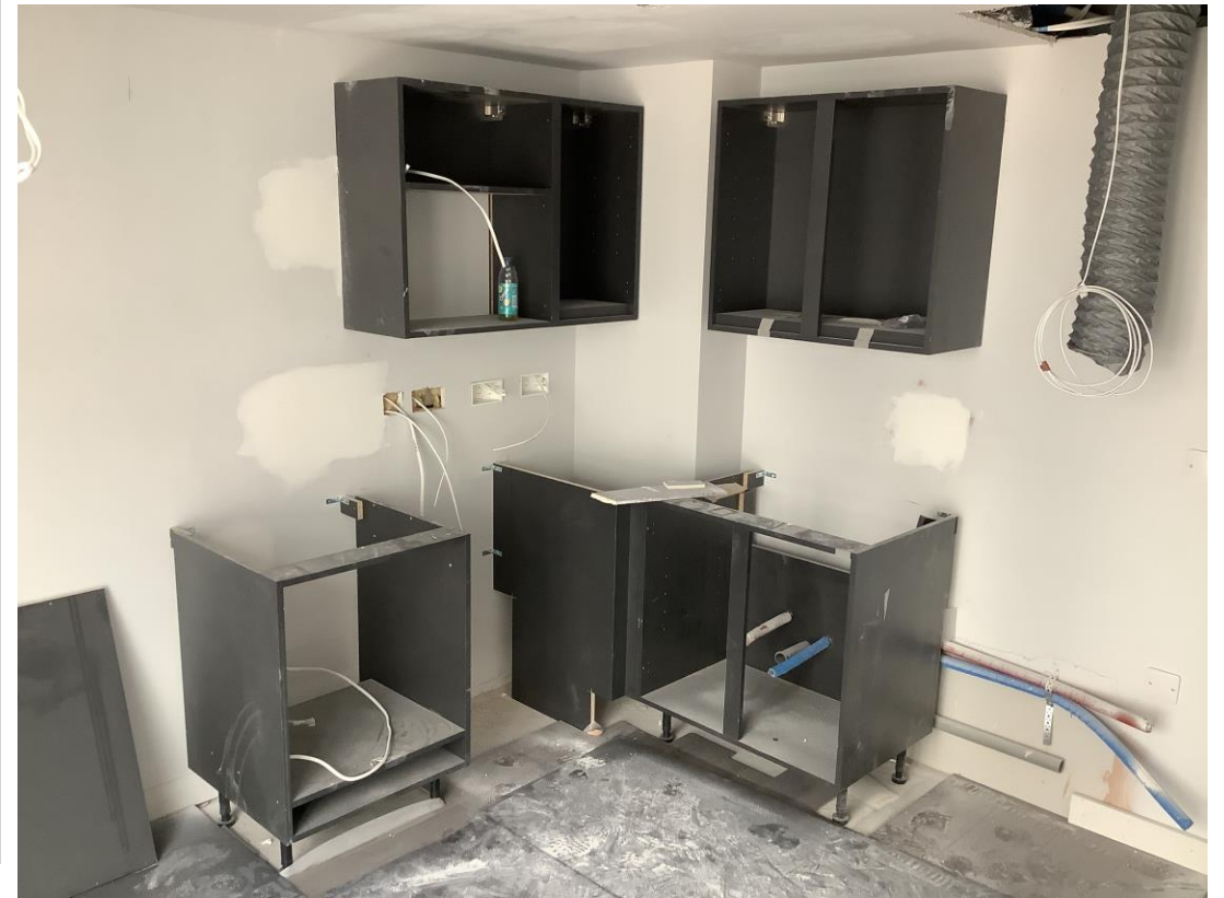
Student wing – Kitchen units on-going
