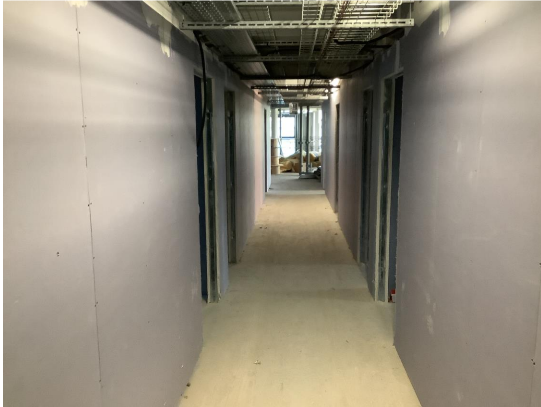
Residential wing – Boarding of partitions on-going
