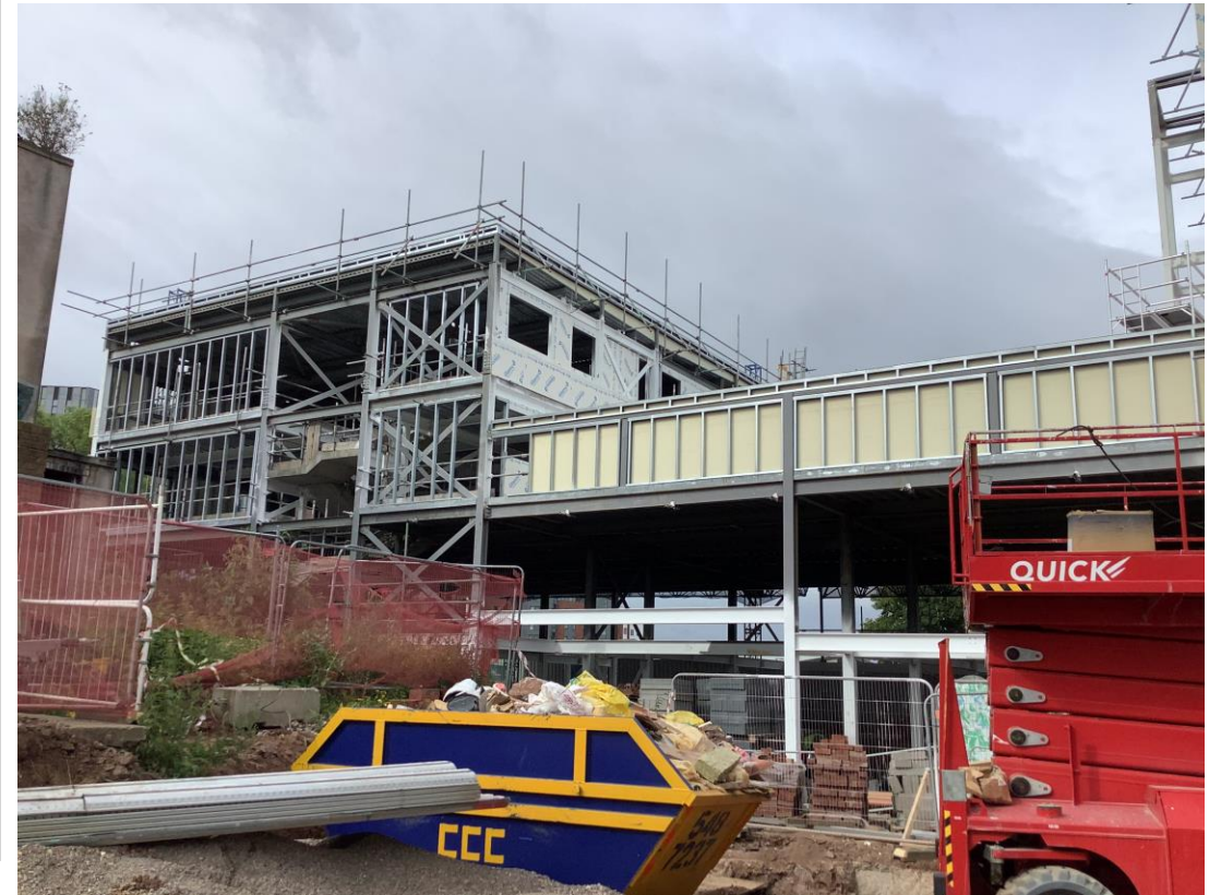
Commercial Block - SFS, weatherboard and windows
