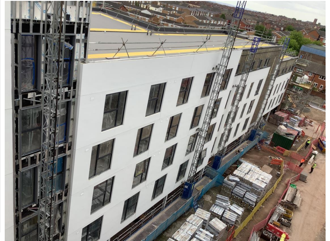
Student Wing – Render application & cladding progress
