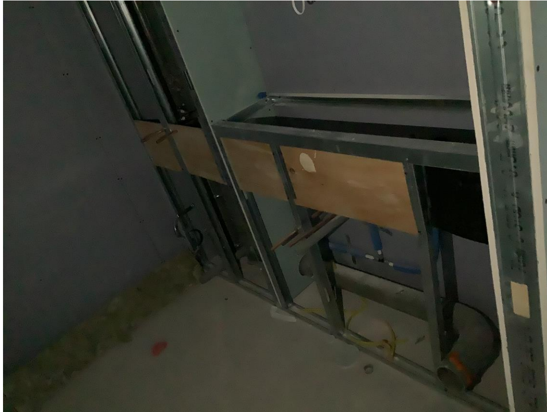
Residential wing – Boarding of recessed drainage installation
