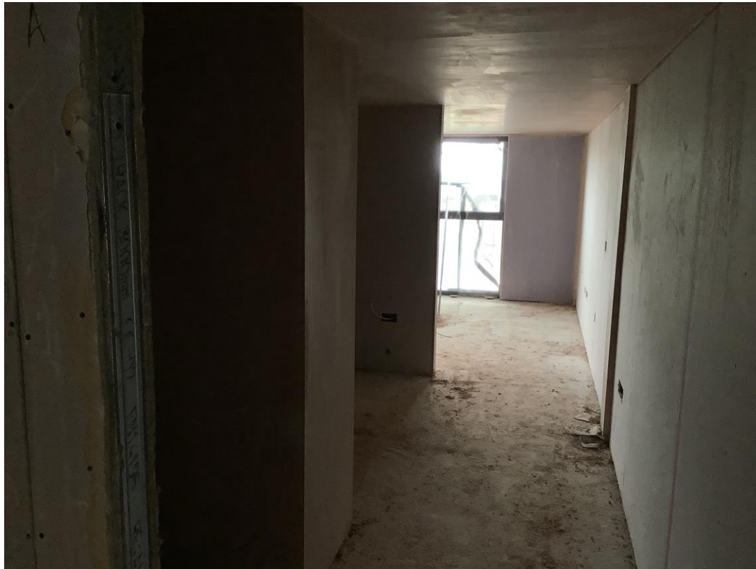
Student wing – Plastering to internal walls
