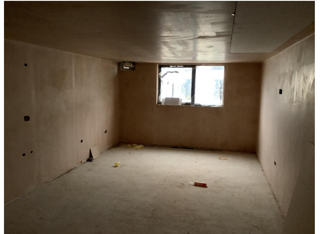
Student wing – Plastering to internal walls
