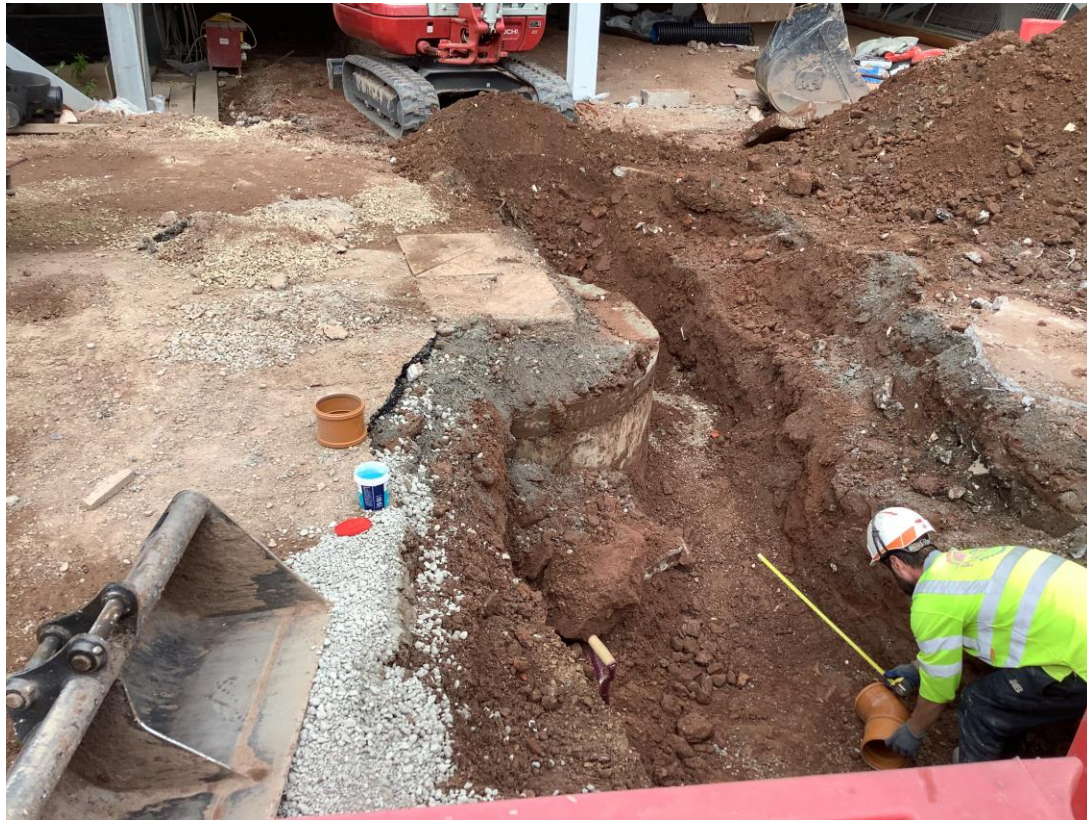
External drainage works
