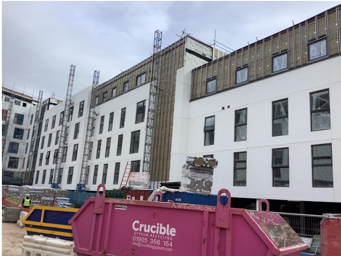
Student Wing – Render application & cladding progress
