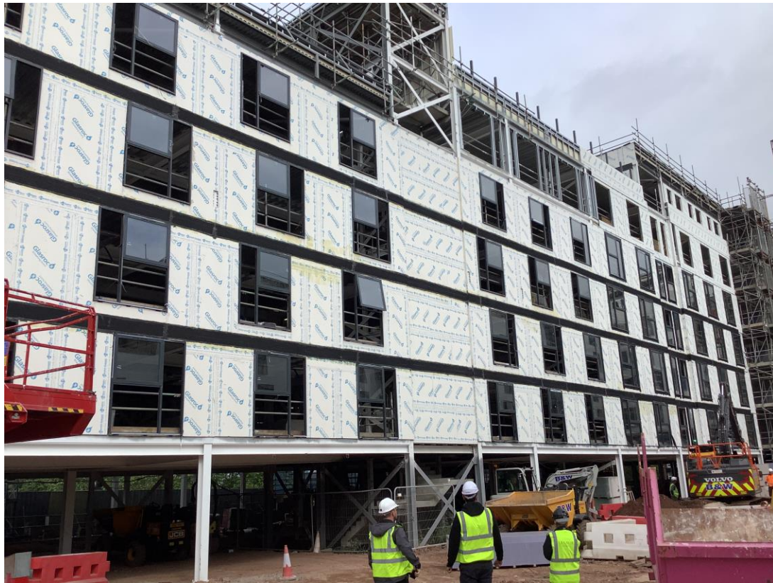
Residential wing – SFS, weatherboard and windows
