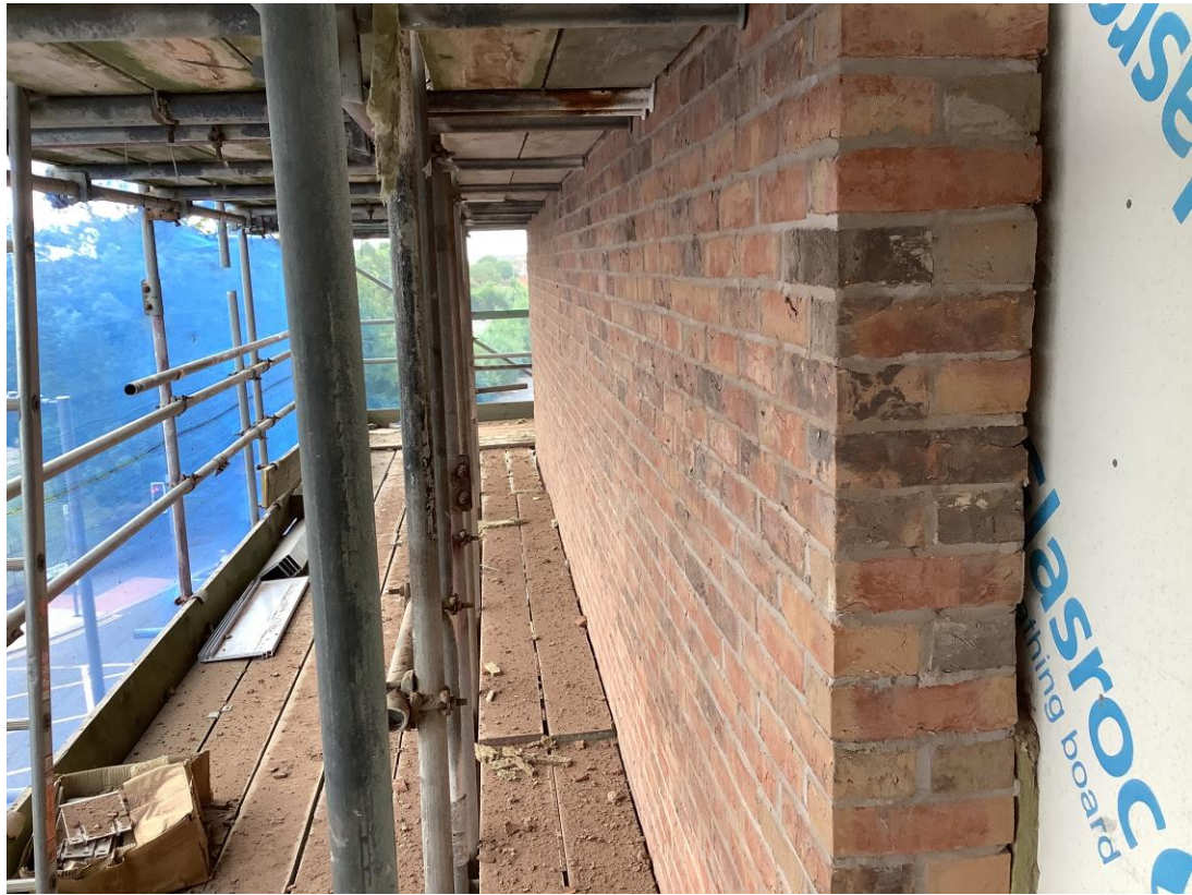
Residential wing – External brickwork on-going
