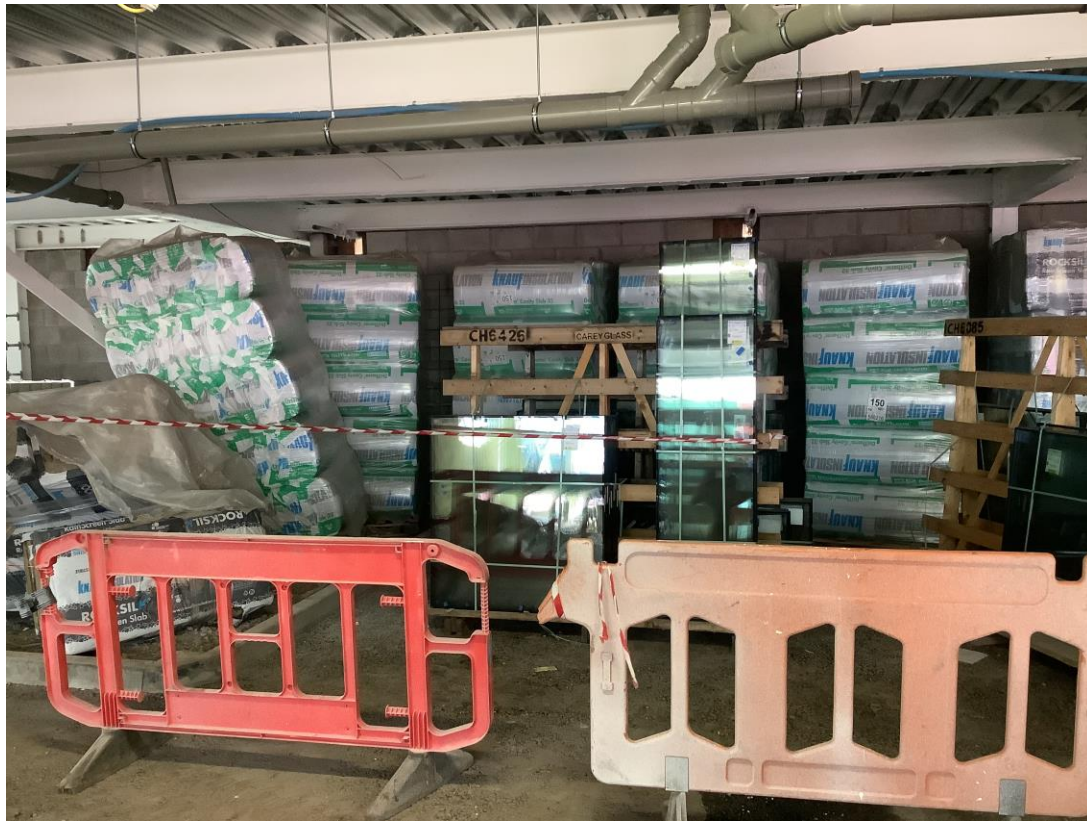
Material storage – Insulation and glazing panels
