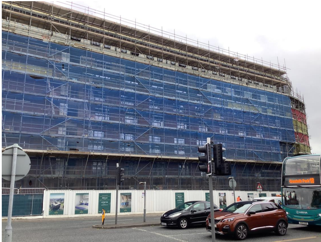
West Derby Road - Site view
