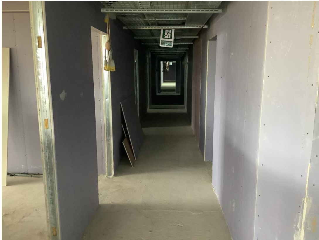
Student wing – Boarding of partitions on-going
