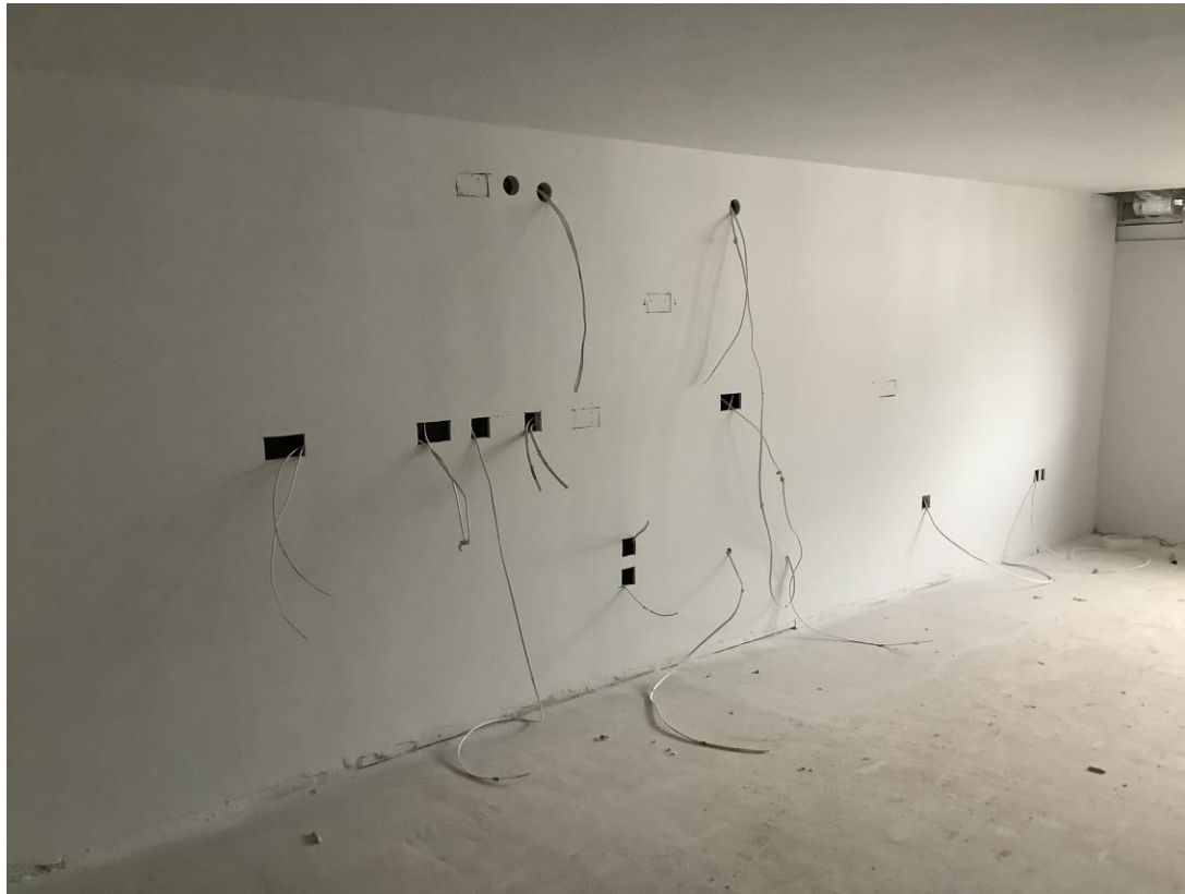
Student wing – 1 st Fix electrical installations
