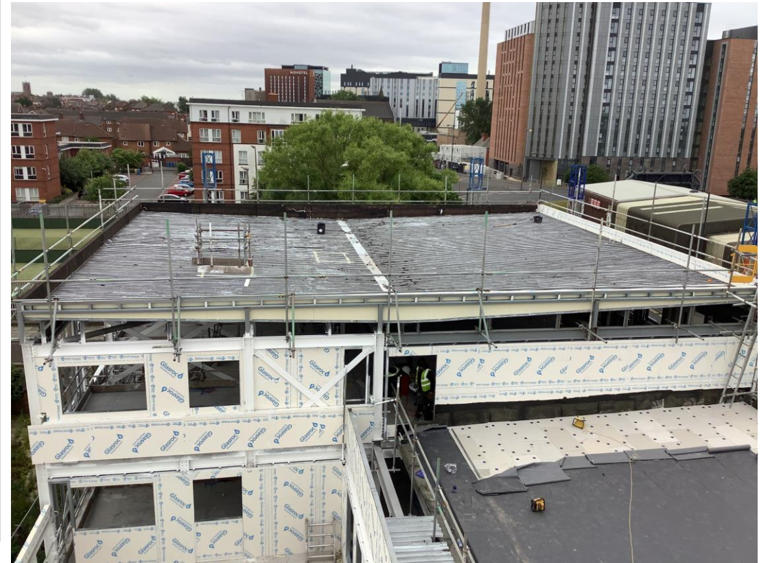
Commercial block – Flat roof construction progress
