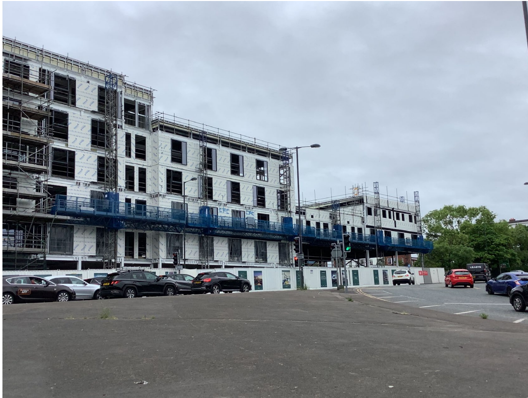
Brunswick Road - Site view
