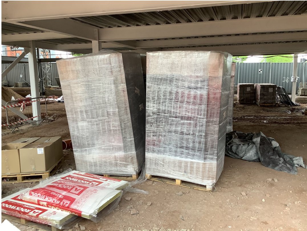
Material storage – Internal lifts
