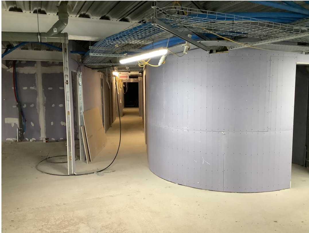
Student wing – Boarding of partitions on-going
