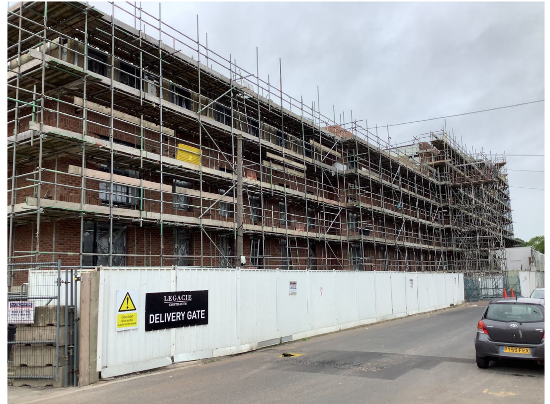
Walker Street - Site view
