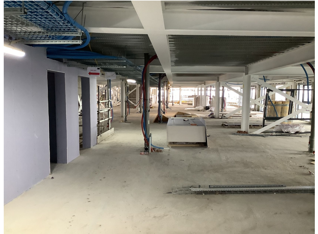
Student wing – Boarding of partitions on-going
