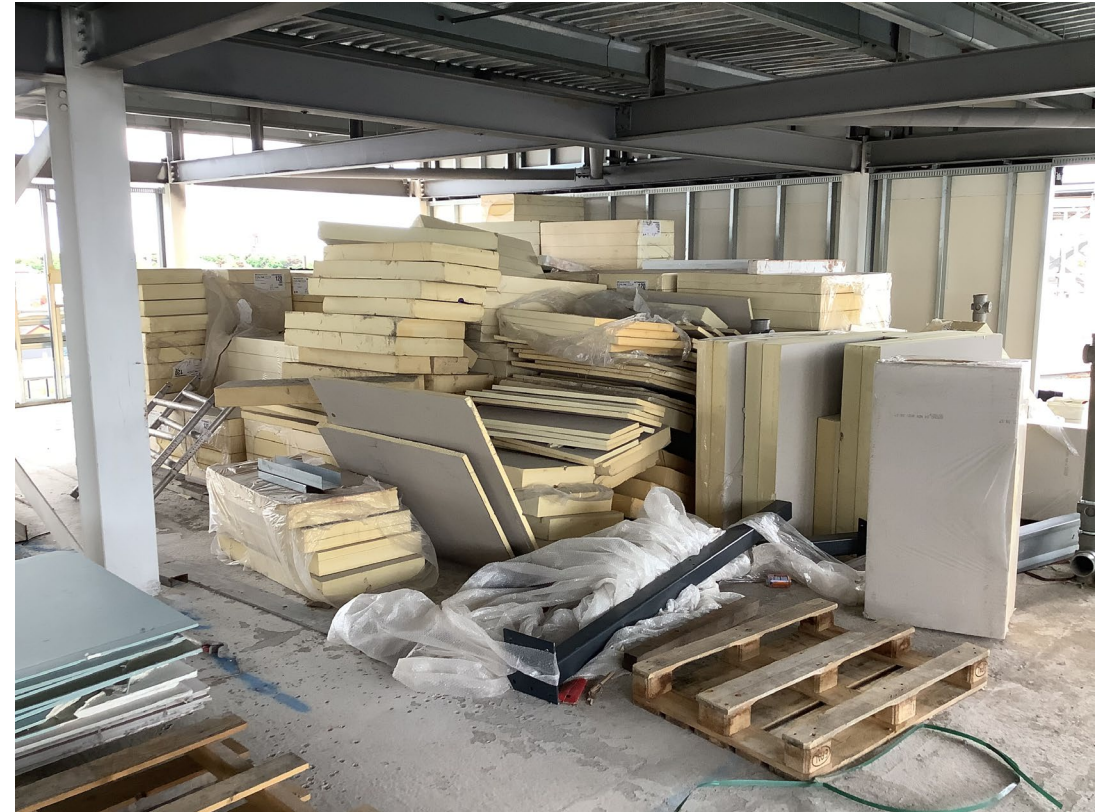
Material storage – Insulation
