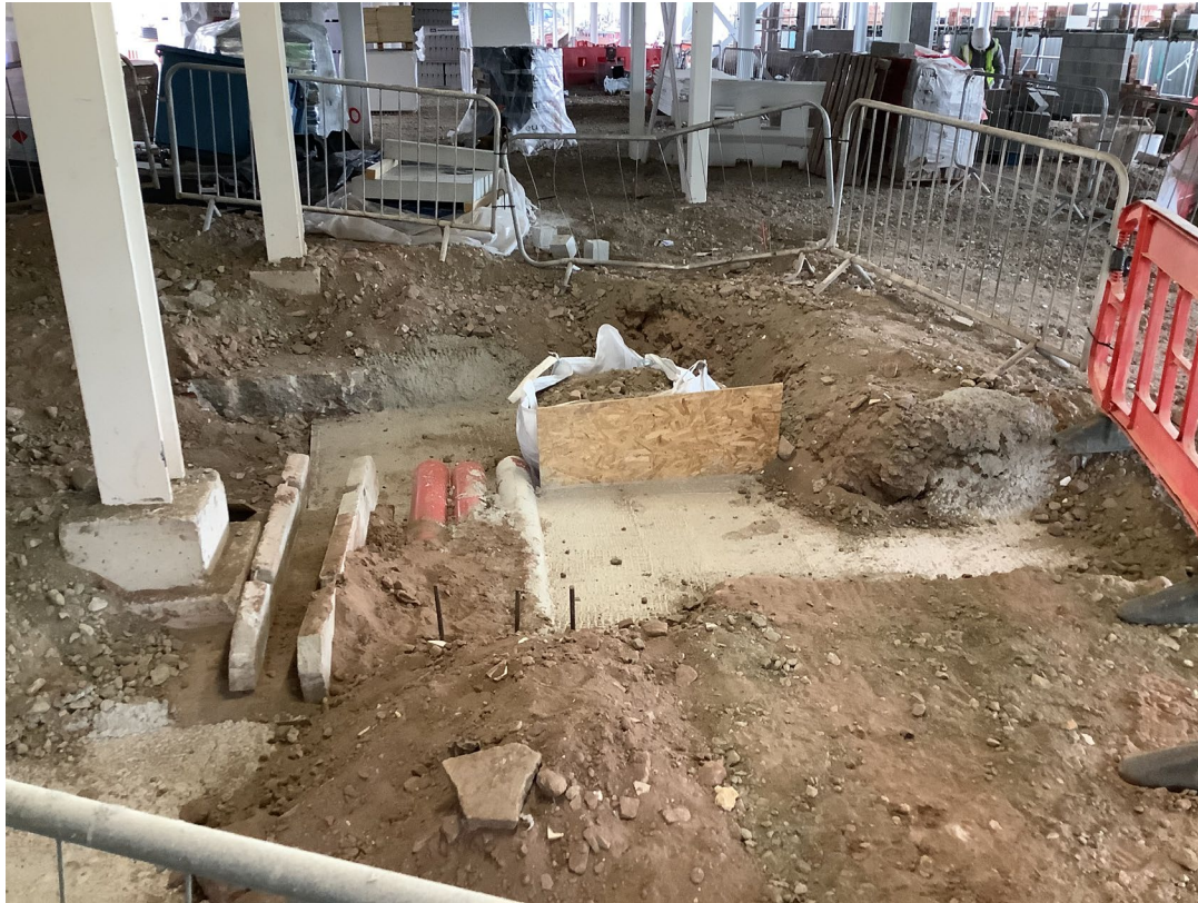
Ground floor - Under ground drainage and ground floor beams
