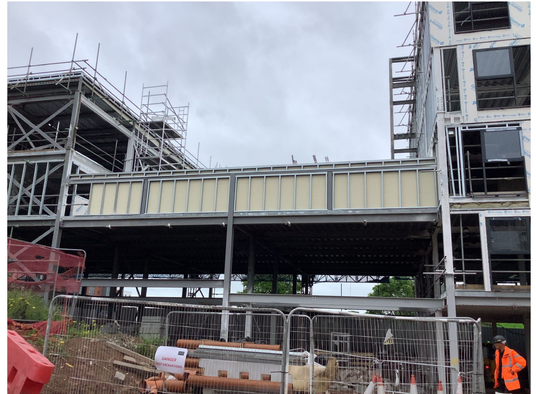
Inner courtyard view – Commercial Block
