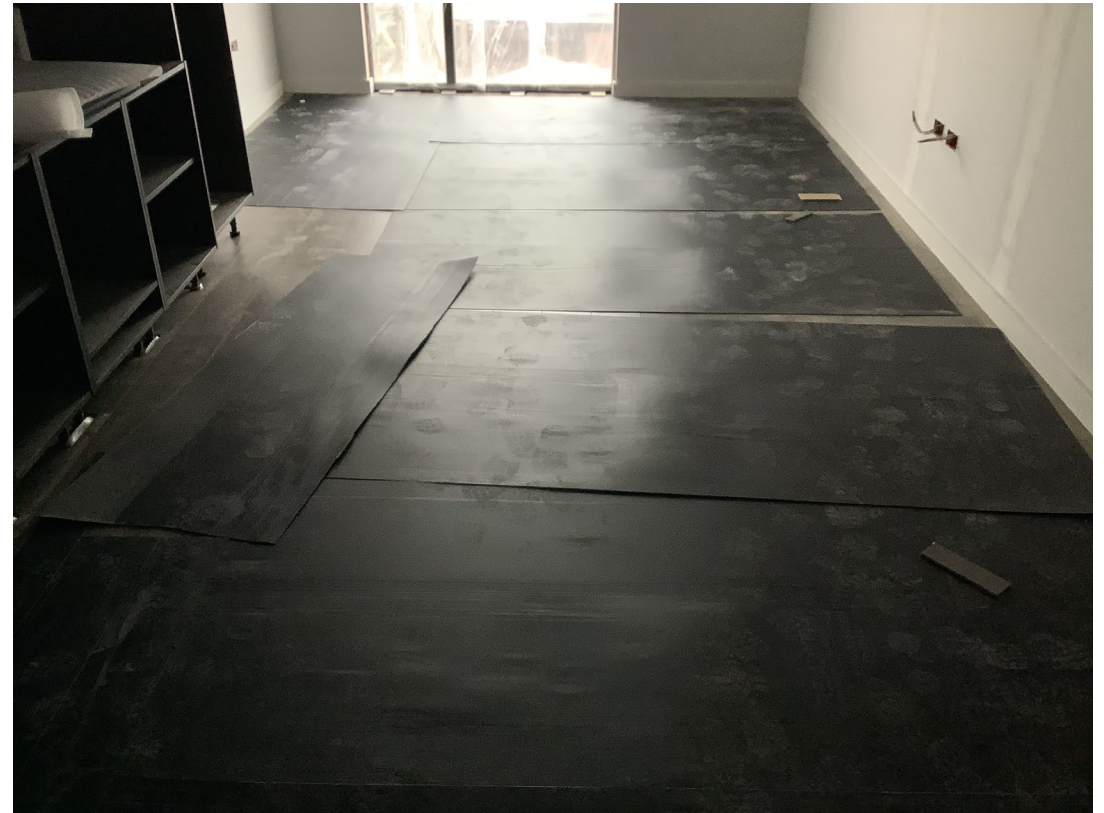
Student wing – Internal floor finishes commenced
