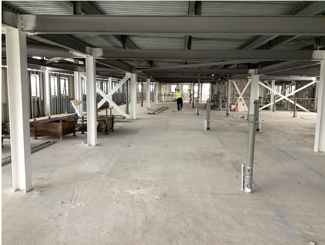
Student wing (Upper Floors) – General record photograph
