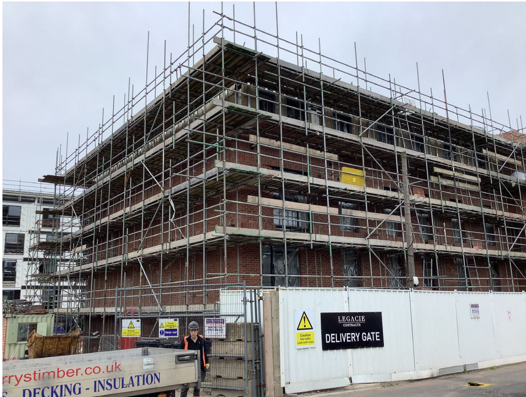
Walker Street - Site view
