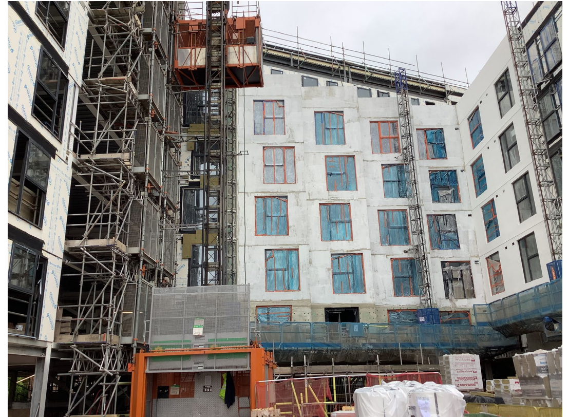
Inner courtyard view – General progress photo
