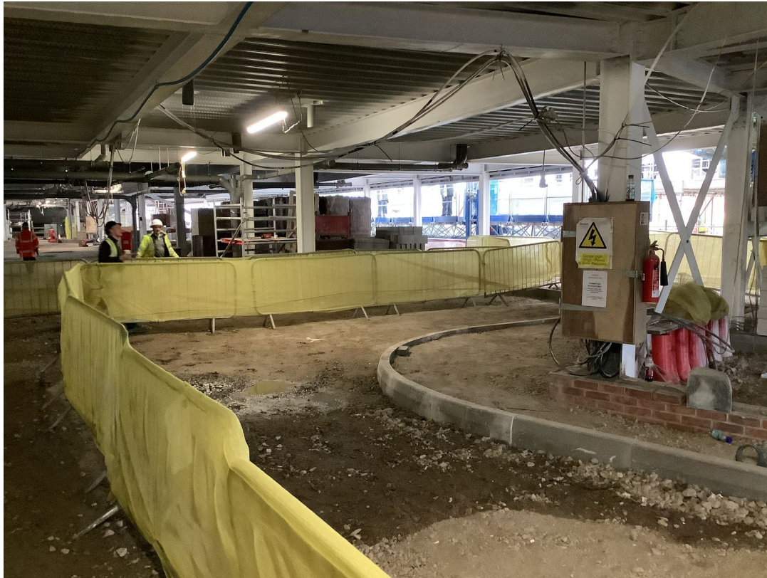
Student wing – Under croft parking progress
