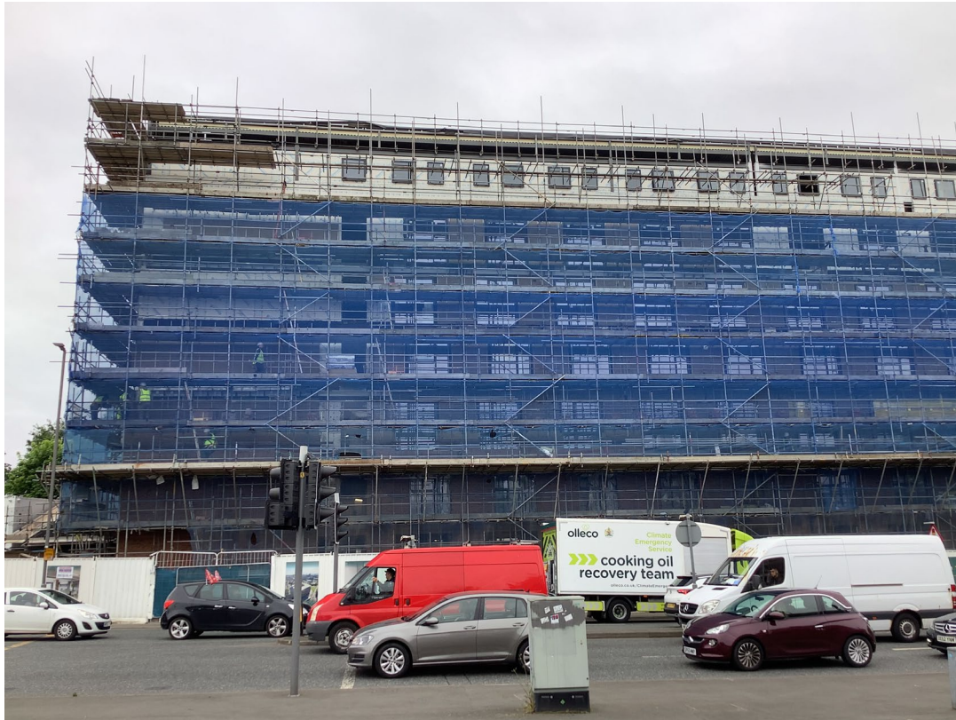
West Derby Road - Site view
