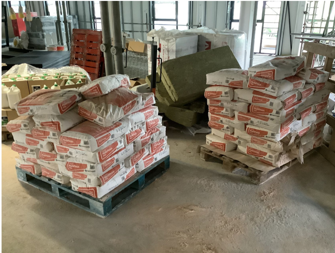
Material storage – Multi-finish plaster
