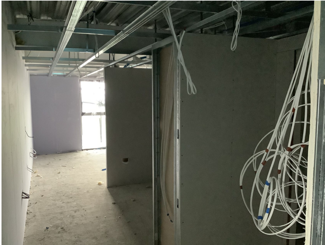
Student wing – Boarding of partitions on-going
