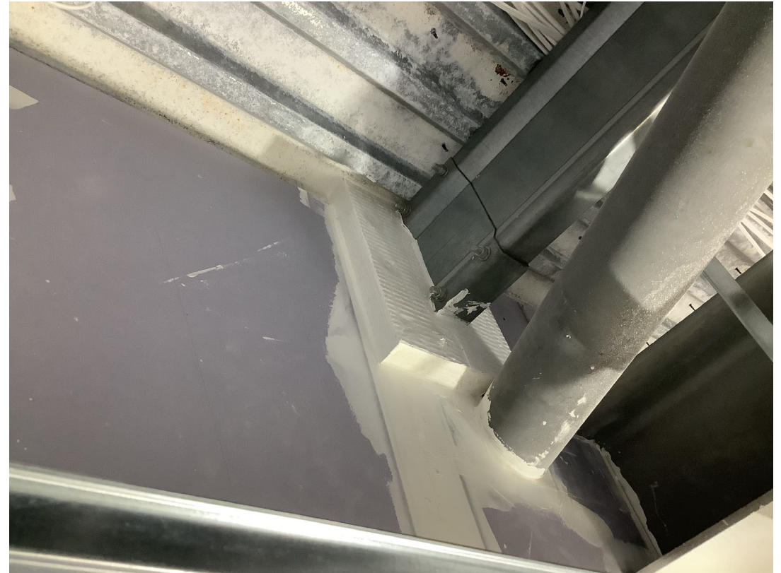
Student wing – Firestopping works on-going
