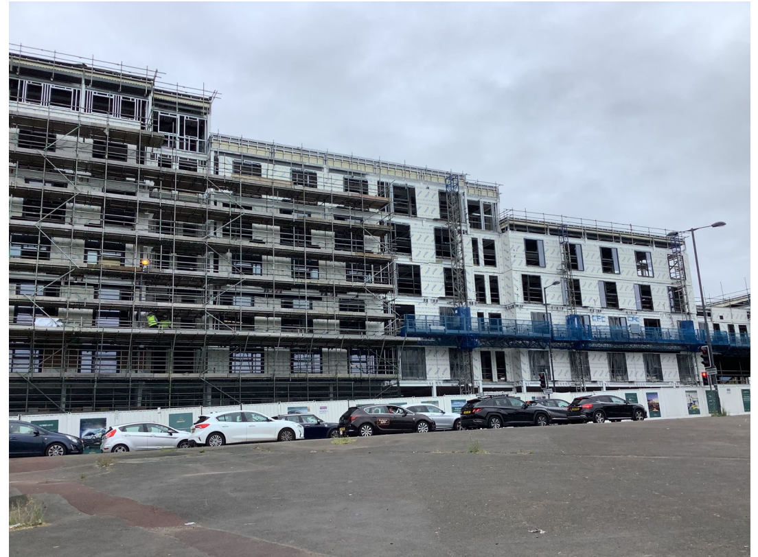
Brunswick Road - Site view
