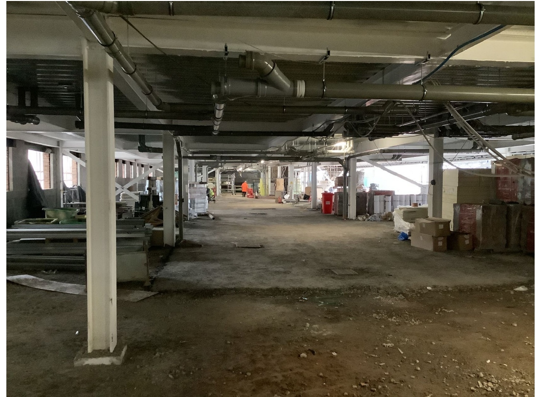
Student wing – Undercroft parking progress
