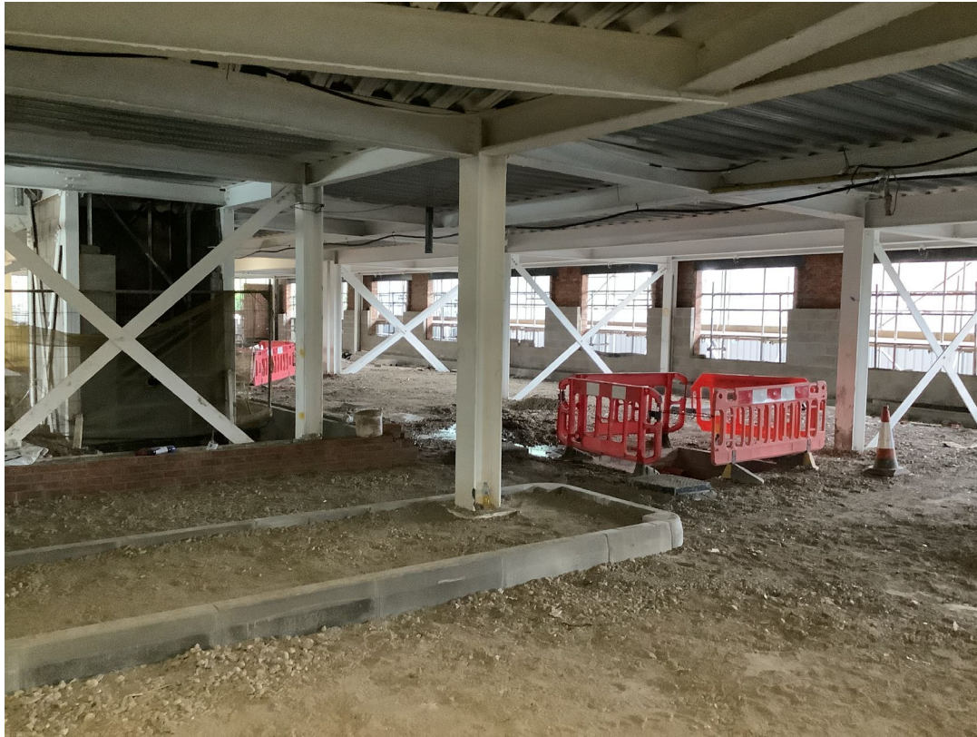
Student wing – Undercroft parking progress
