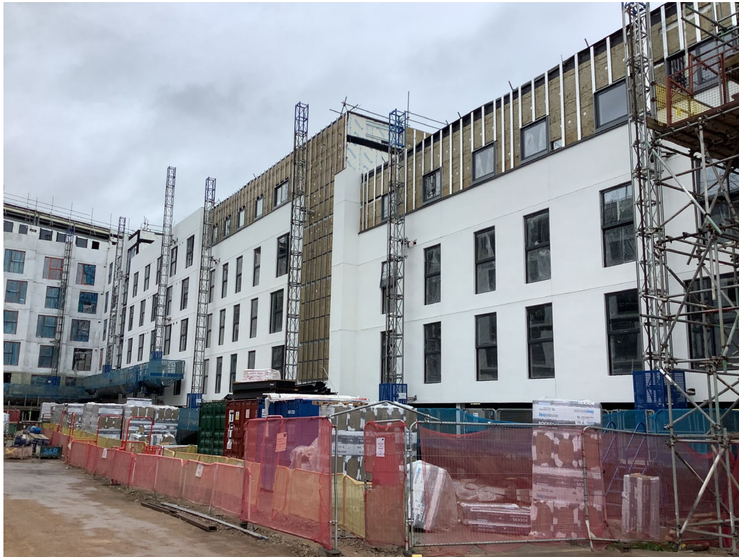
Inner courtyard view – Render application & cladding progress
