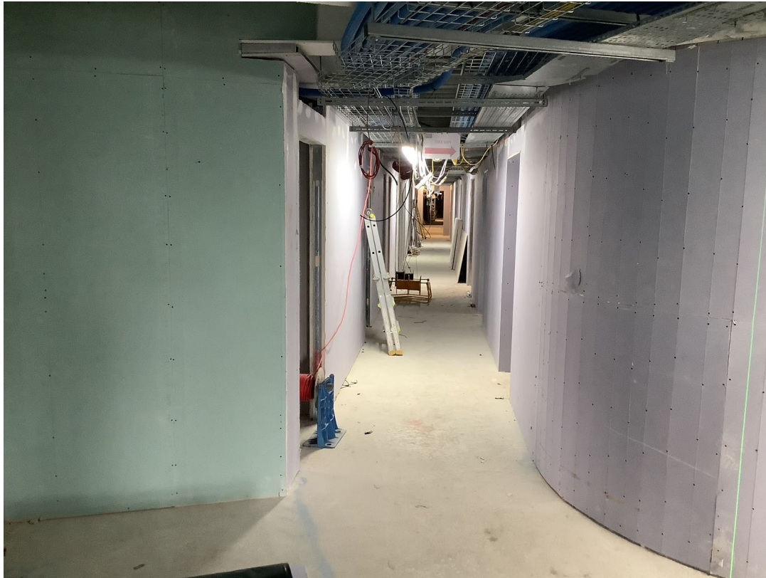
Student wing – Boarding of partitions on-going
