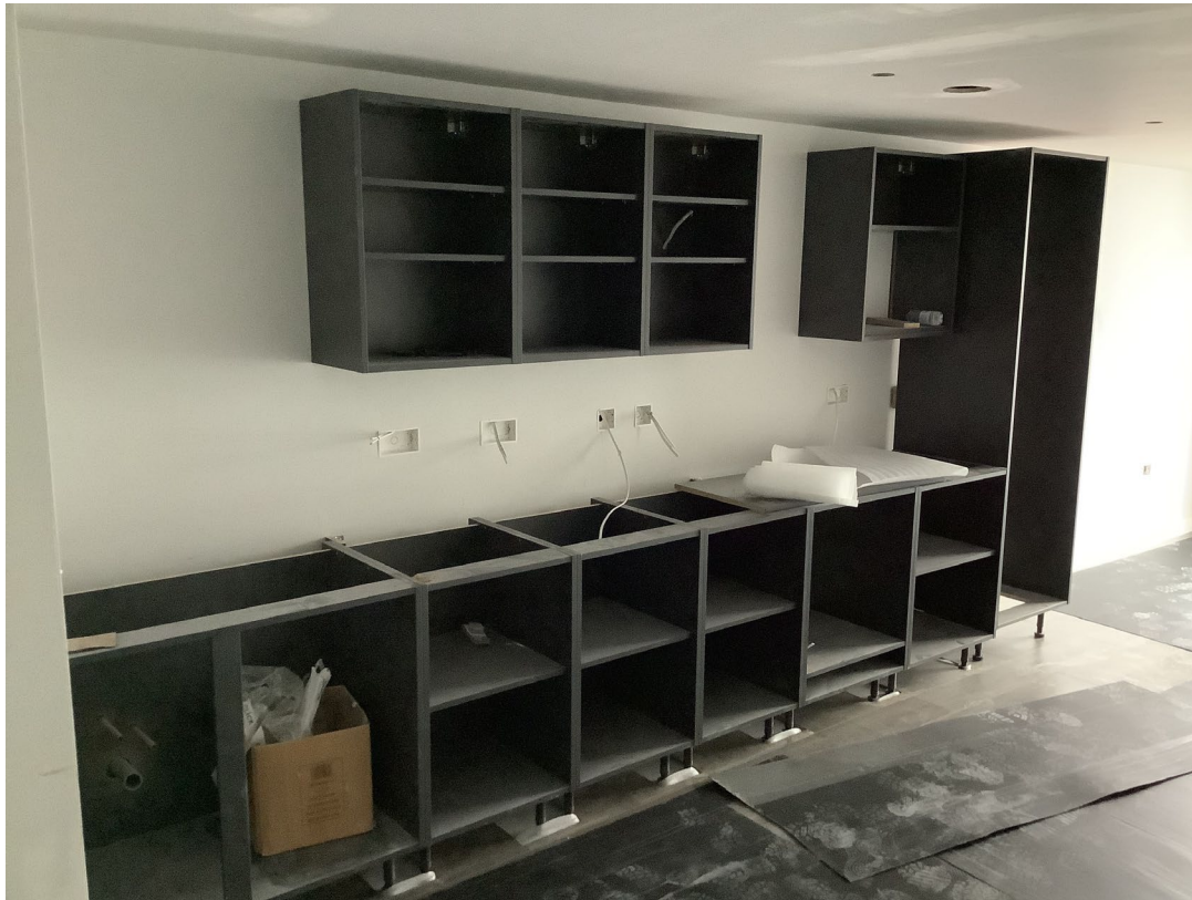
Student wing – Kitchen units commenced
