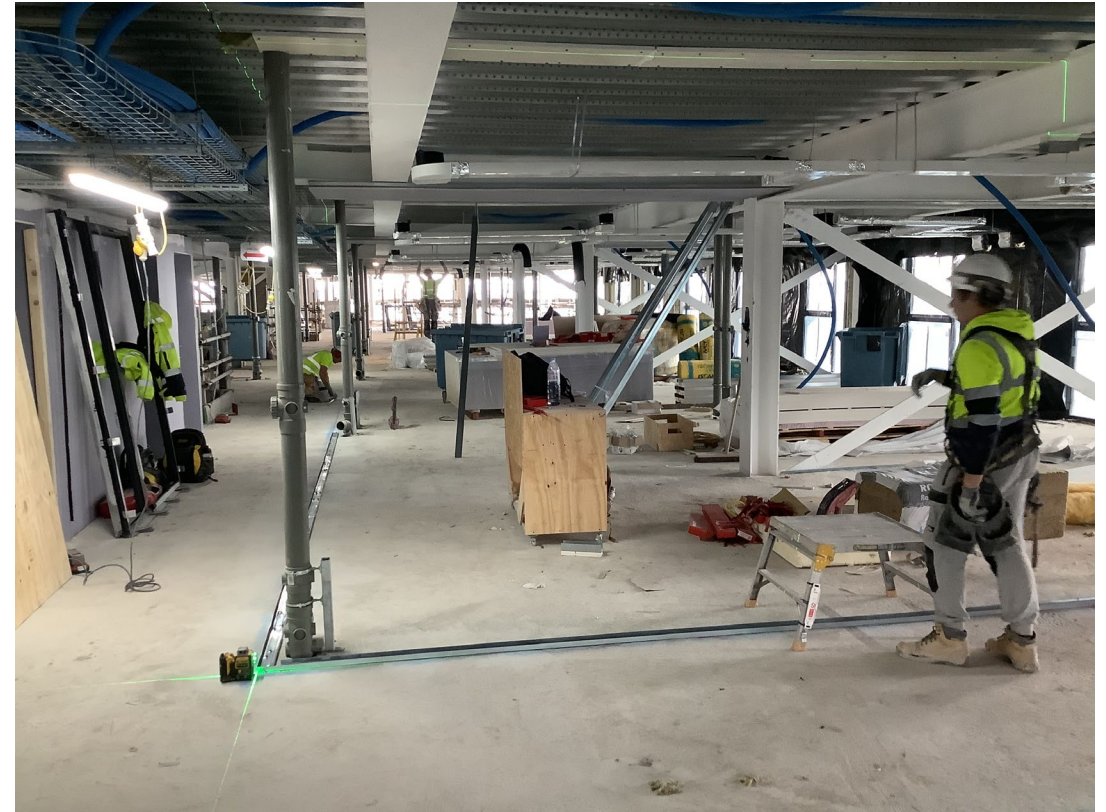
Student wing – Boarding of partitions on-going
