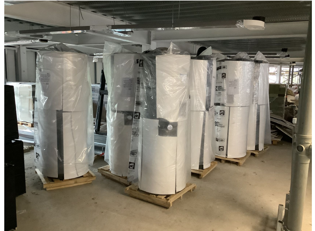
Material storage – KERS energy recovery units
