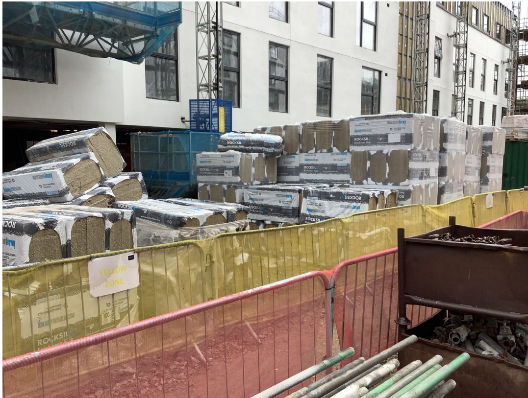
Material storage – Insulation
