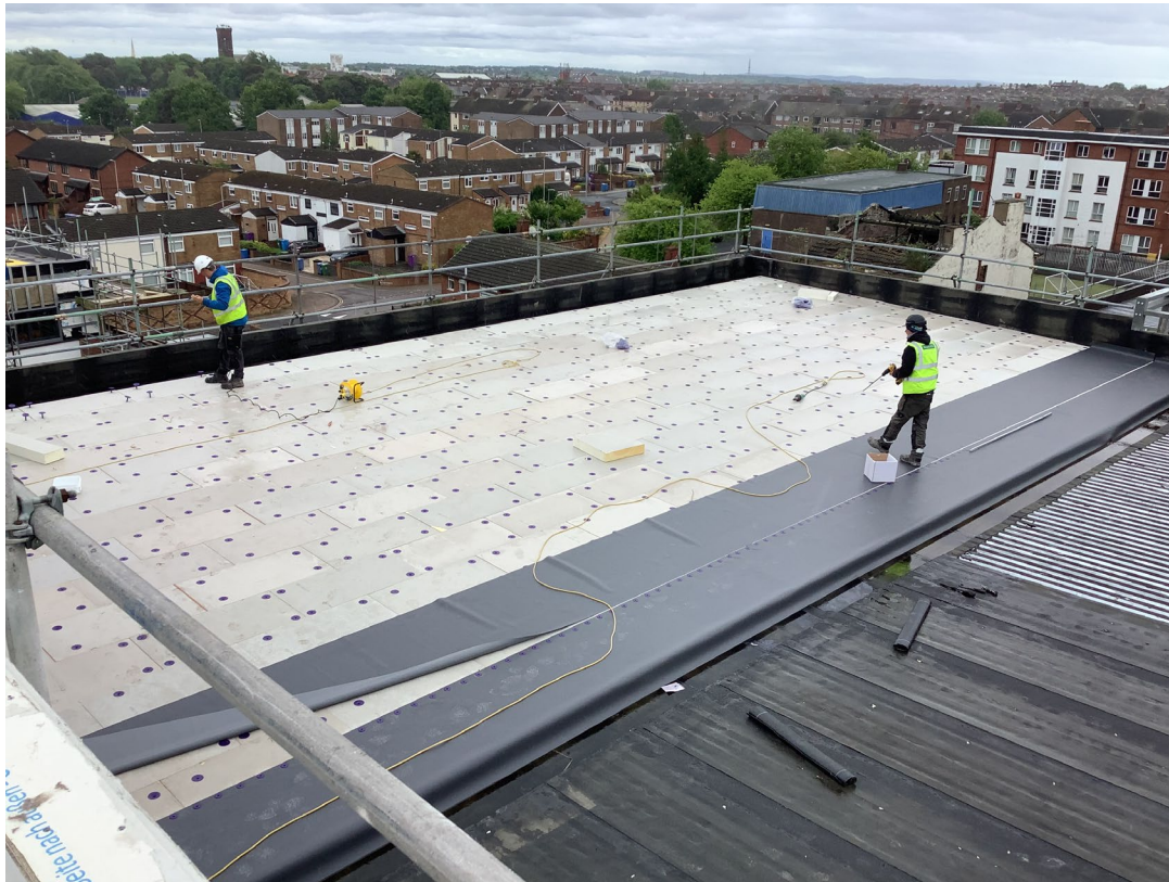
Residential wing – Flat roof coverings progress
