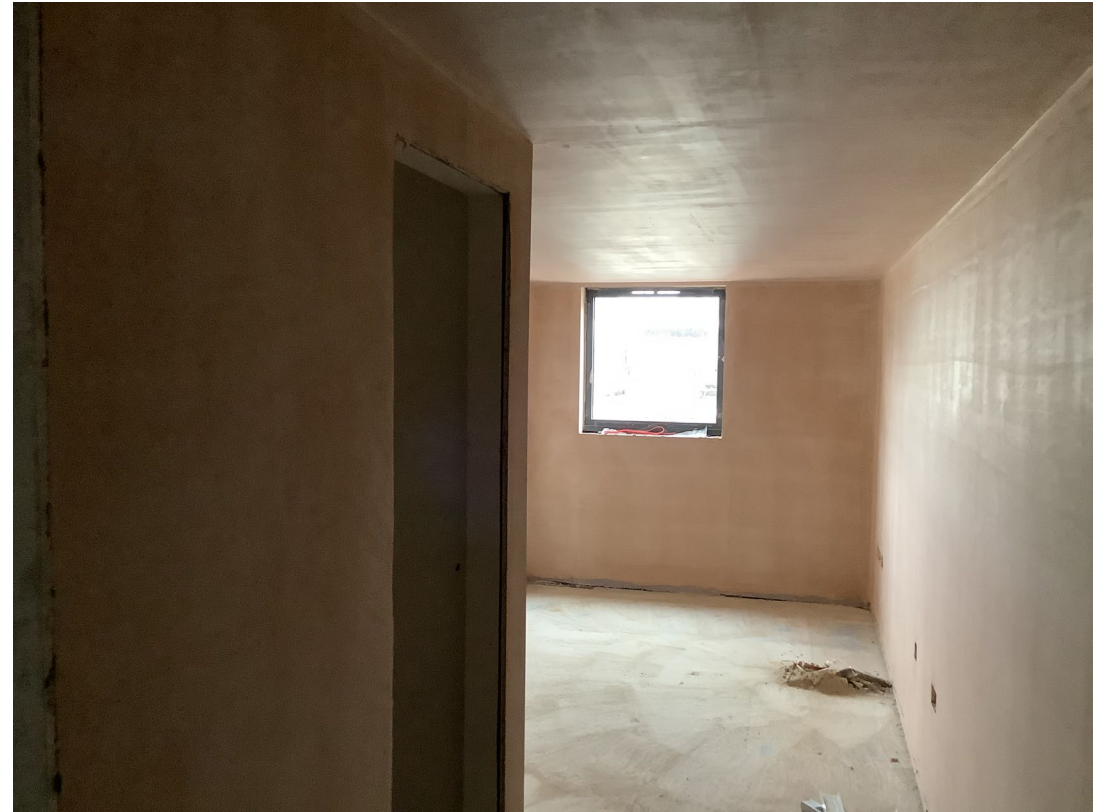
Student wing – Drylining & plasterwork
