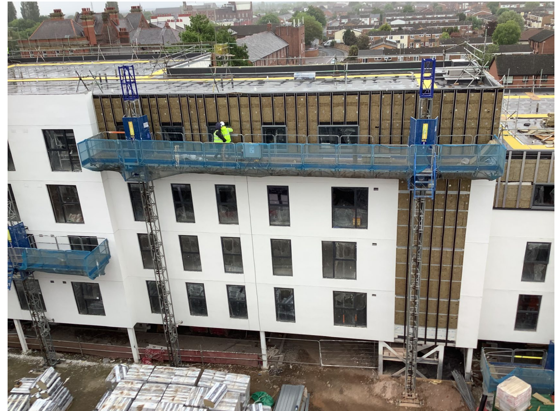
Inner courtyard view – Render application & cladding progress
