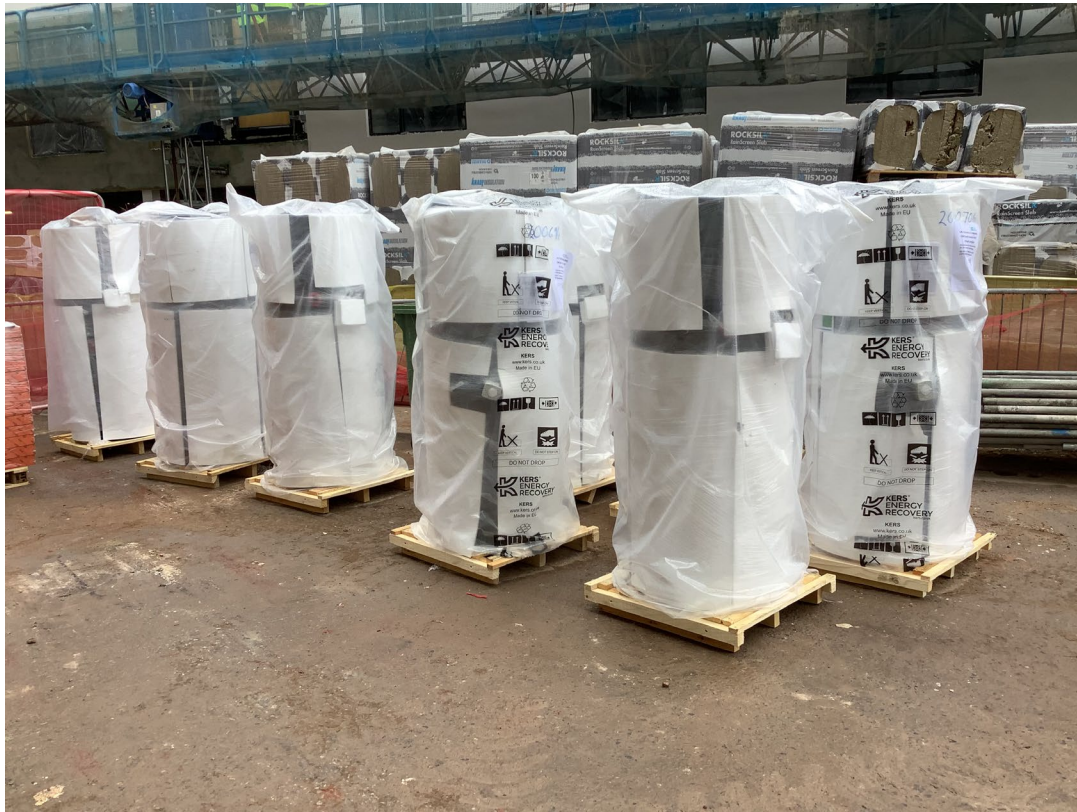
Material storage – KERS energy recovery units
