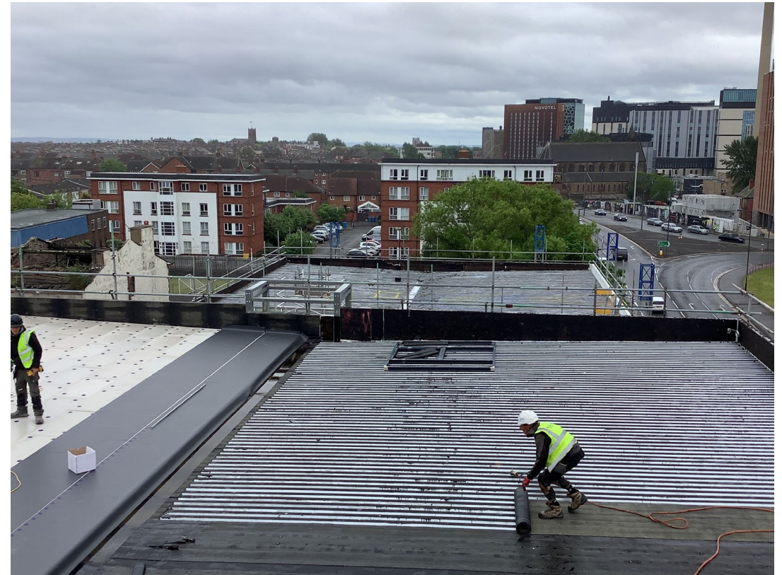
Residential wing – Flat roof coverings progress
