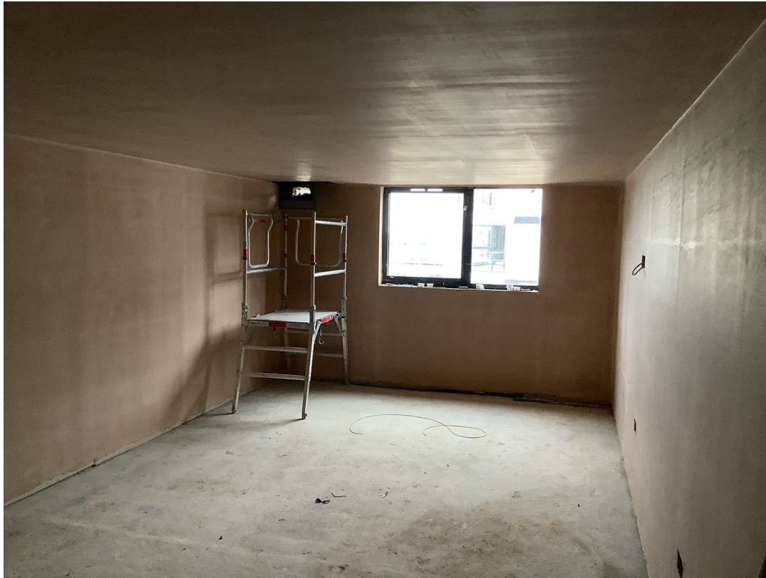
Student wing – Drylining & plasterwork
