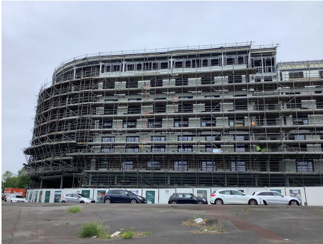
Brunswick Road - Site view
