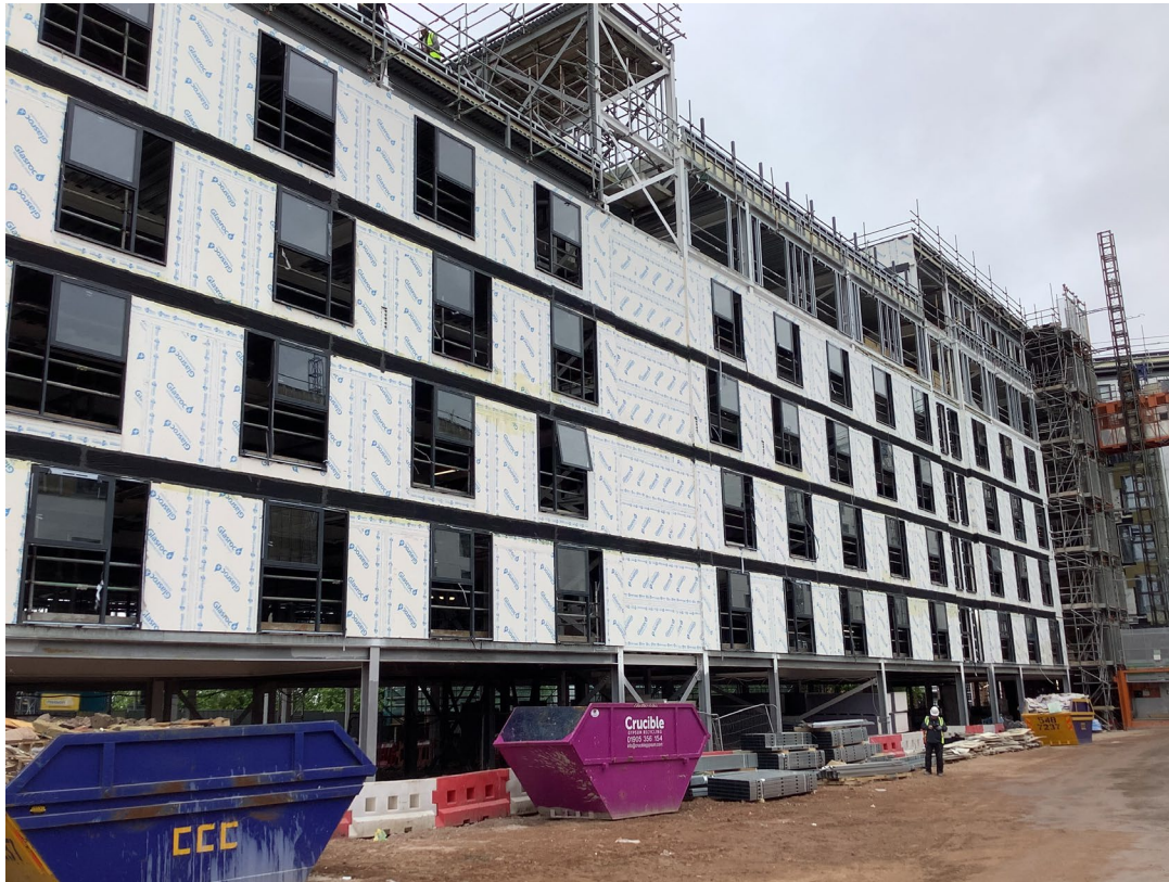
Residential wing - Steel frame structure, SFS & weatherboard and windows
