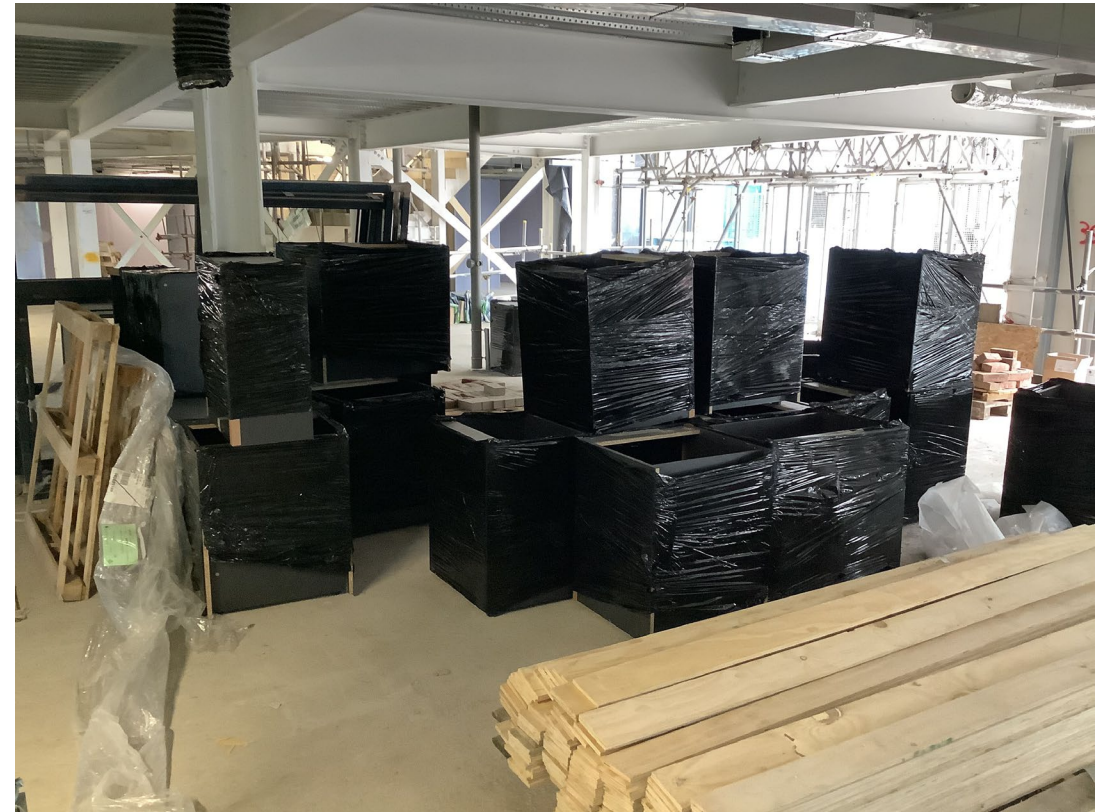
Material storage – Kitchen units
