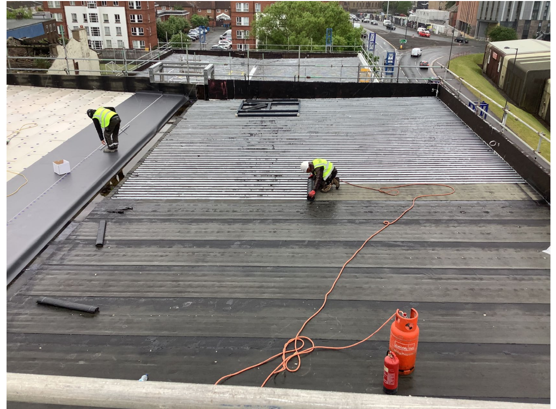
Residential wing – Flat roof coverings progress
