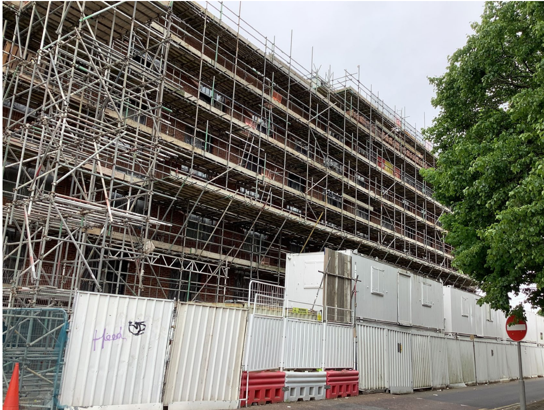
Walker Street - Site view
