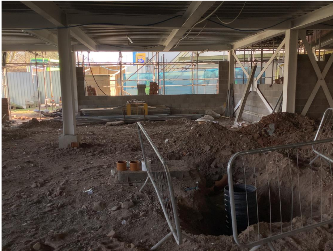
Ground floor - Facing blockwork
