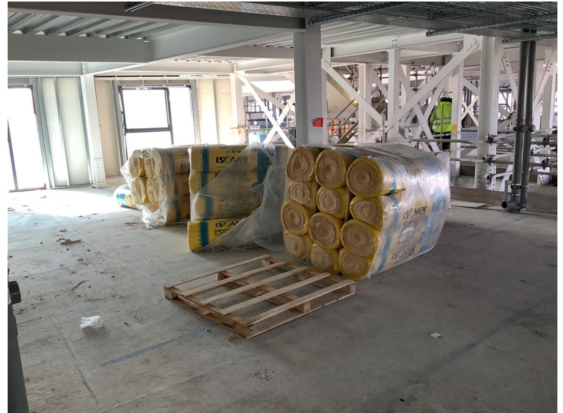
Material storage - Internal insulation
