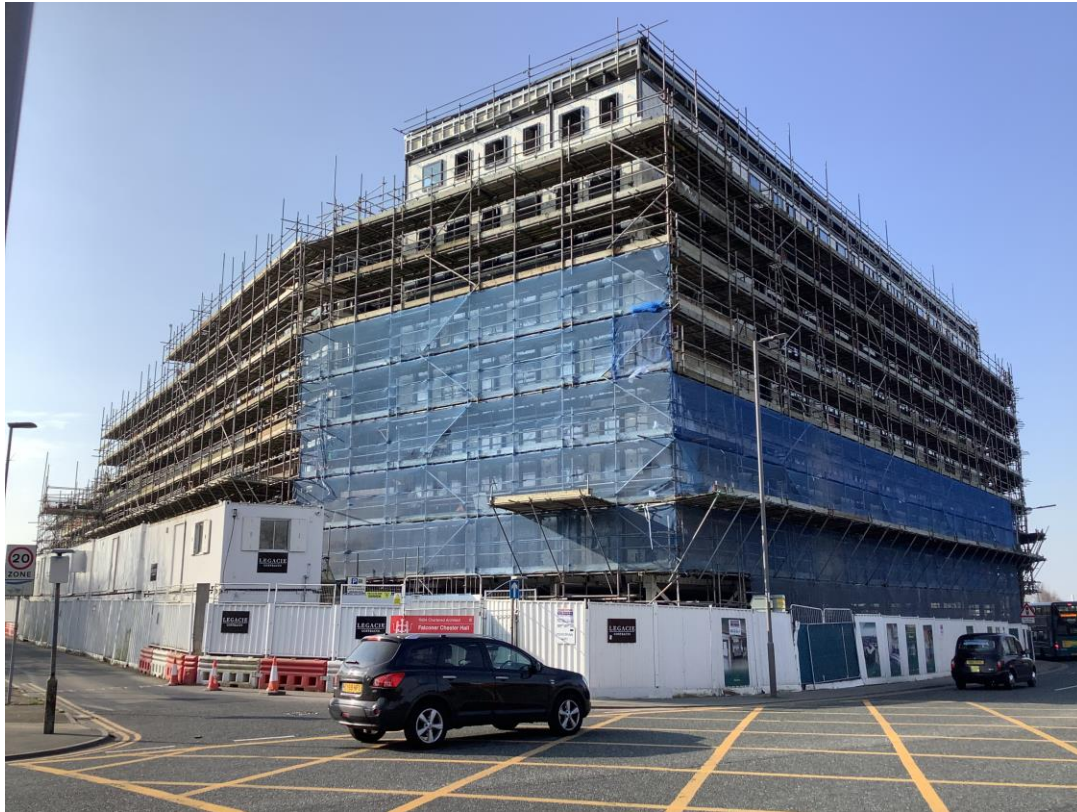
West Derby Road - Site view
