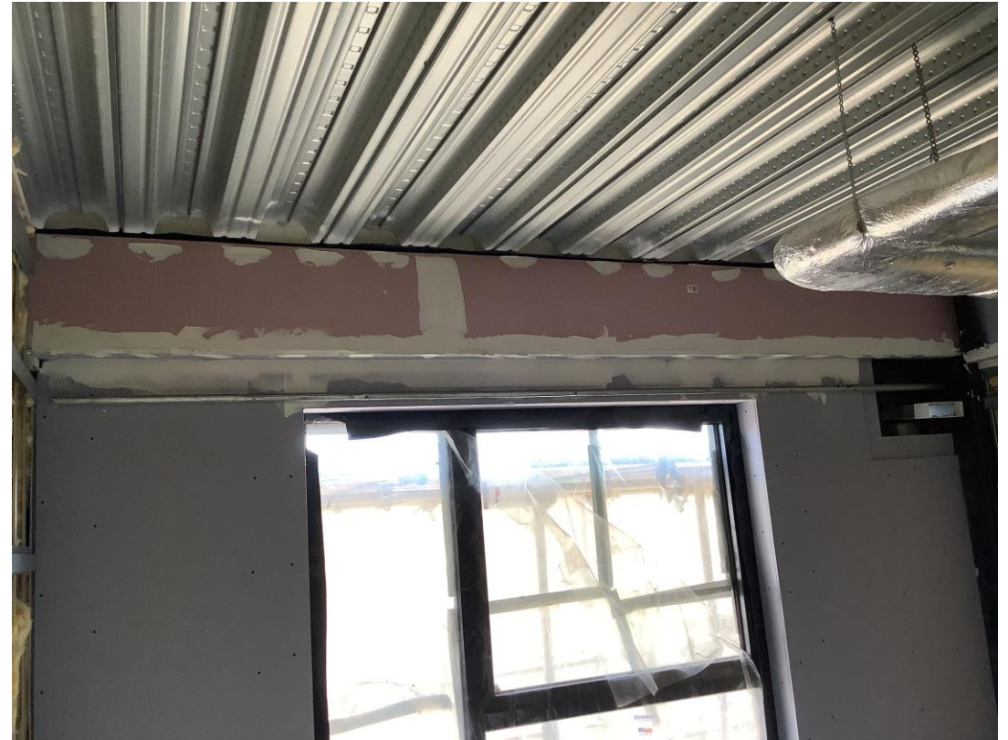
Student wing - Internal fireline plasterboard boxing in
