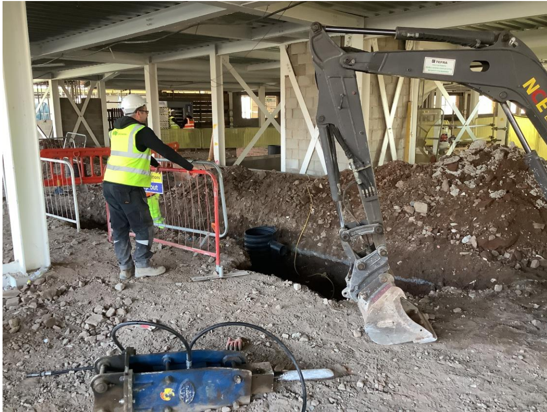
Ground floor trenching works for drainage
