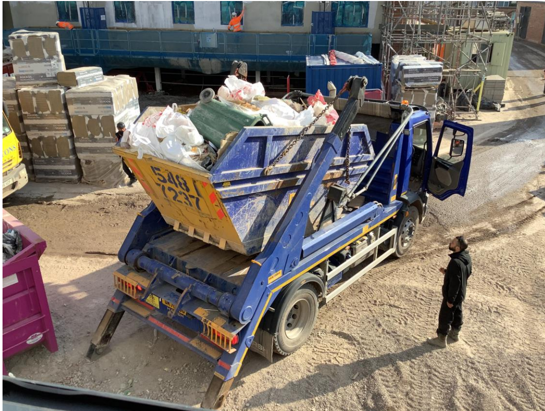
General site activity - Waste removal
