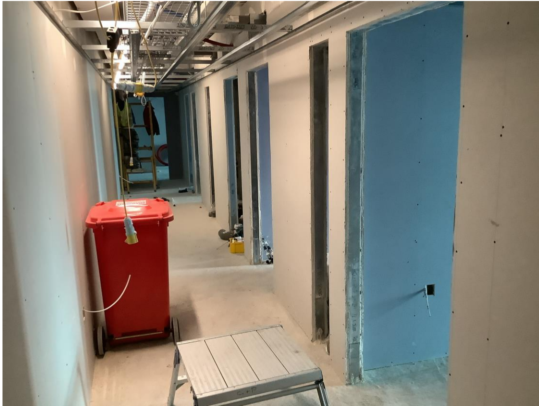
Student wing - Cluster rooms, general view
