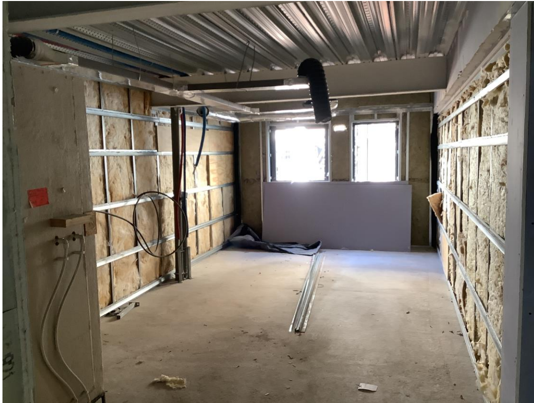
Student wing - Internal metal partitions & insulation
