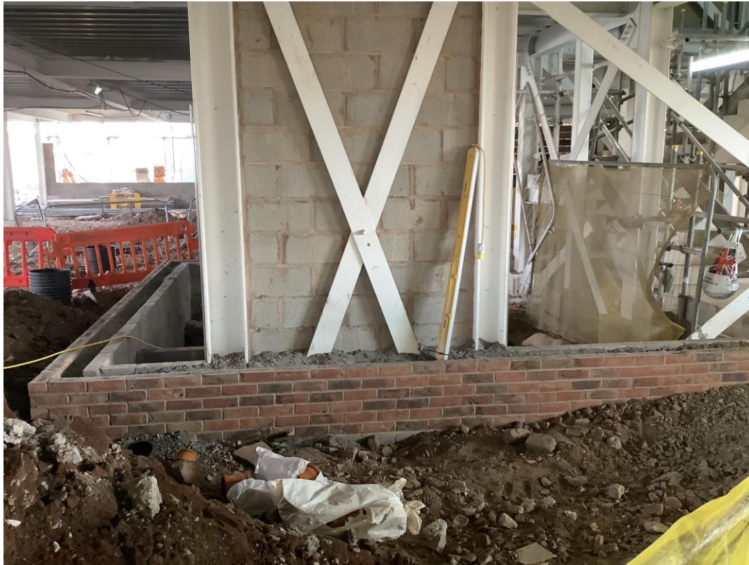
Student wing - Block and brickwork to stair core
