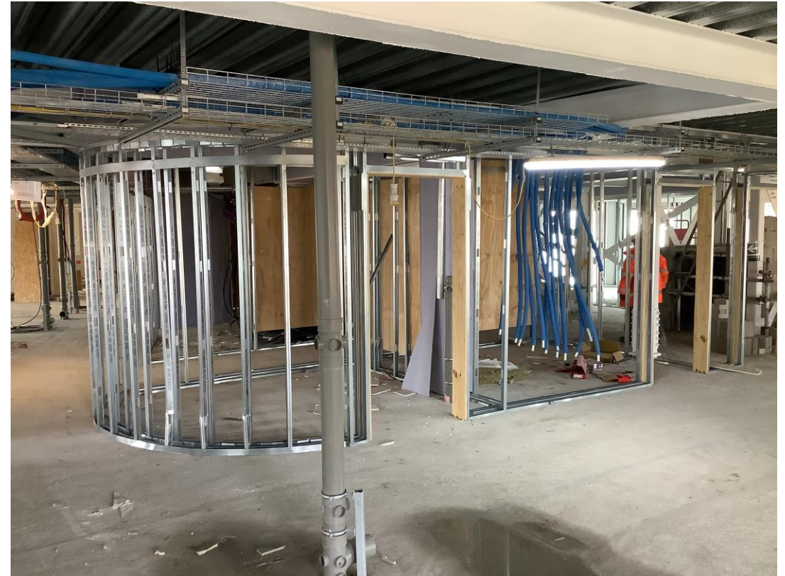
Student wing - Internal metal partitions
