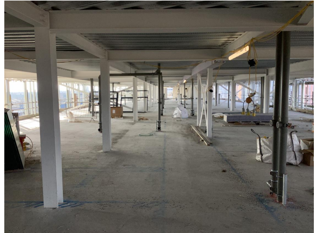
Residential wing - General progress to upper floor
