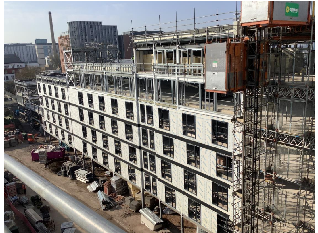
Student wing view - Steel frame structure, SFS & weatherboard and windows
