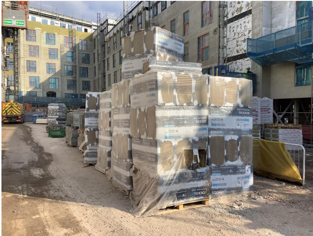
Material storage - External insulation
