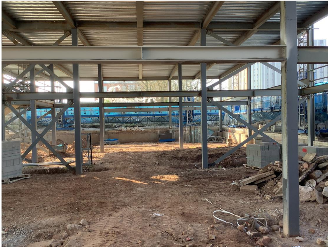
Commercial block - Intumescent coating progress
