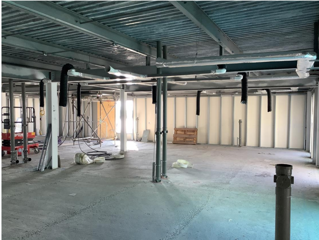
Student wing - General progress to upper floor
