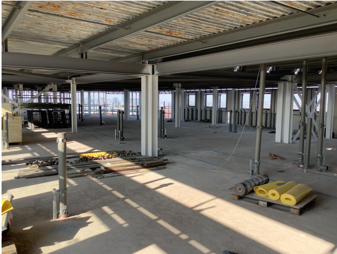
Student wing - General progress to upper floor
