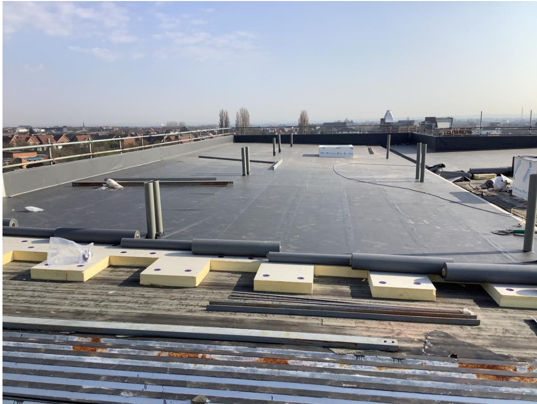
Residential wing - Flat roof coverings
