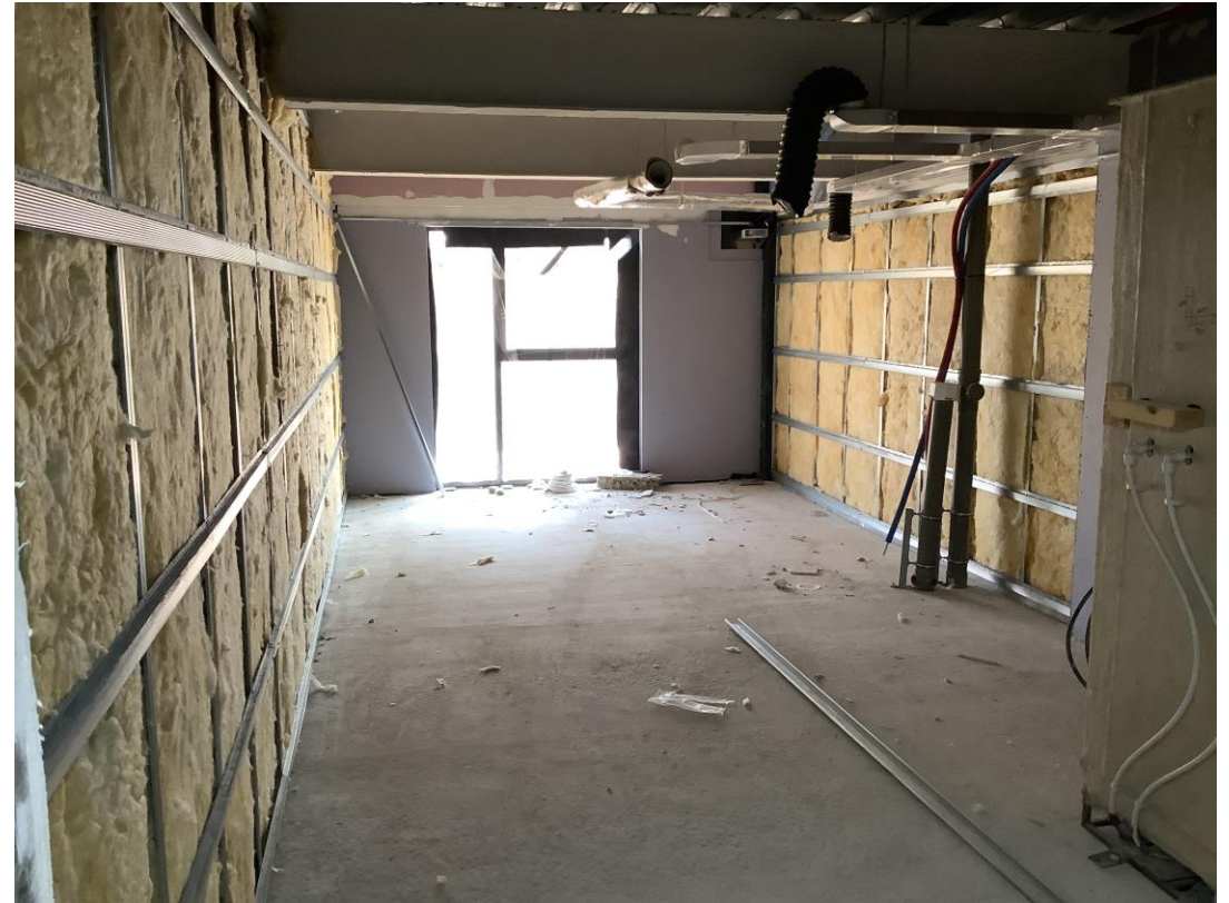
Student wing - Internal metal partitions, insulation & plasterboard
