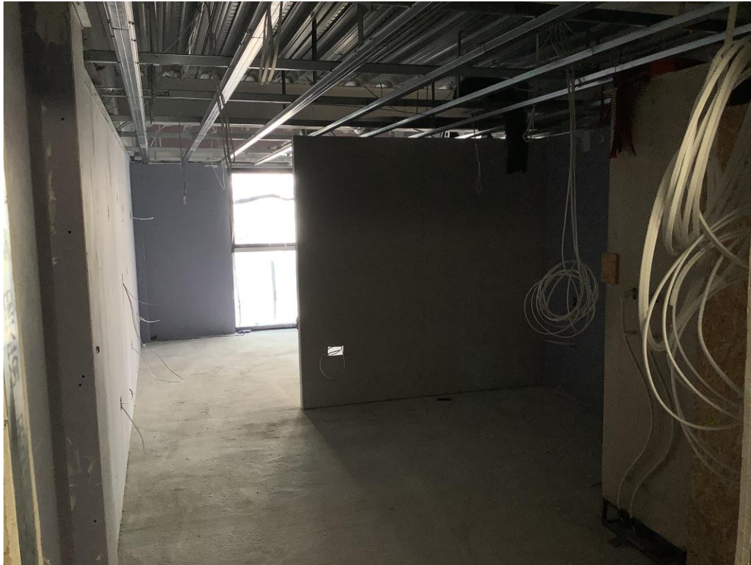
Student wing - Internal metal partitions, plasterboard & metal frame ceiling
