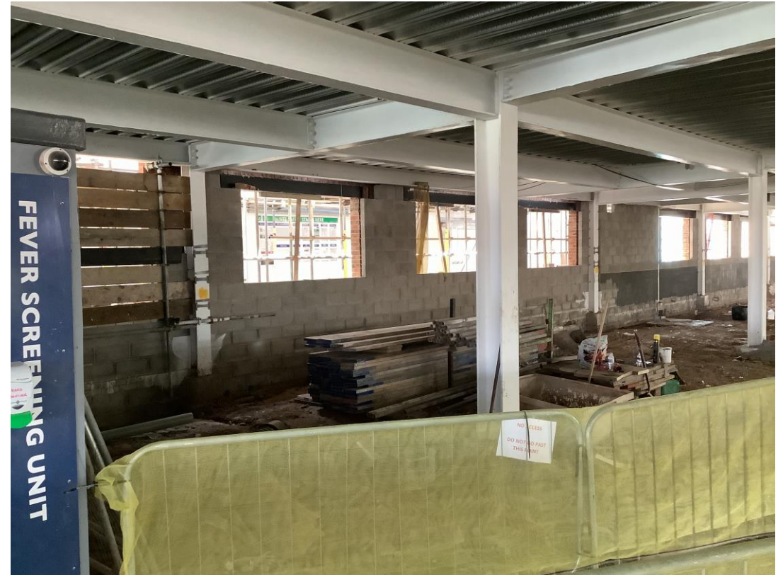
Ground floor - Facing blockwork
