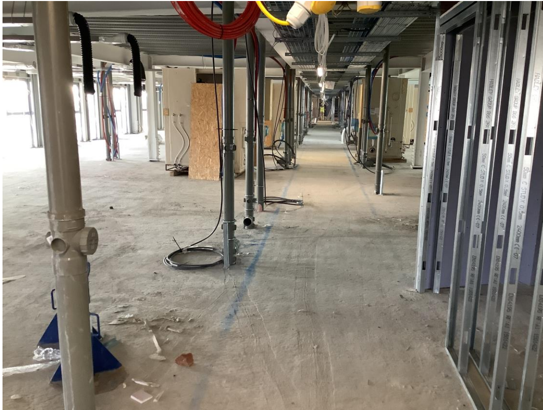
Student wing - Setting out of partitions
