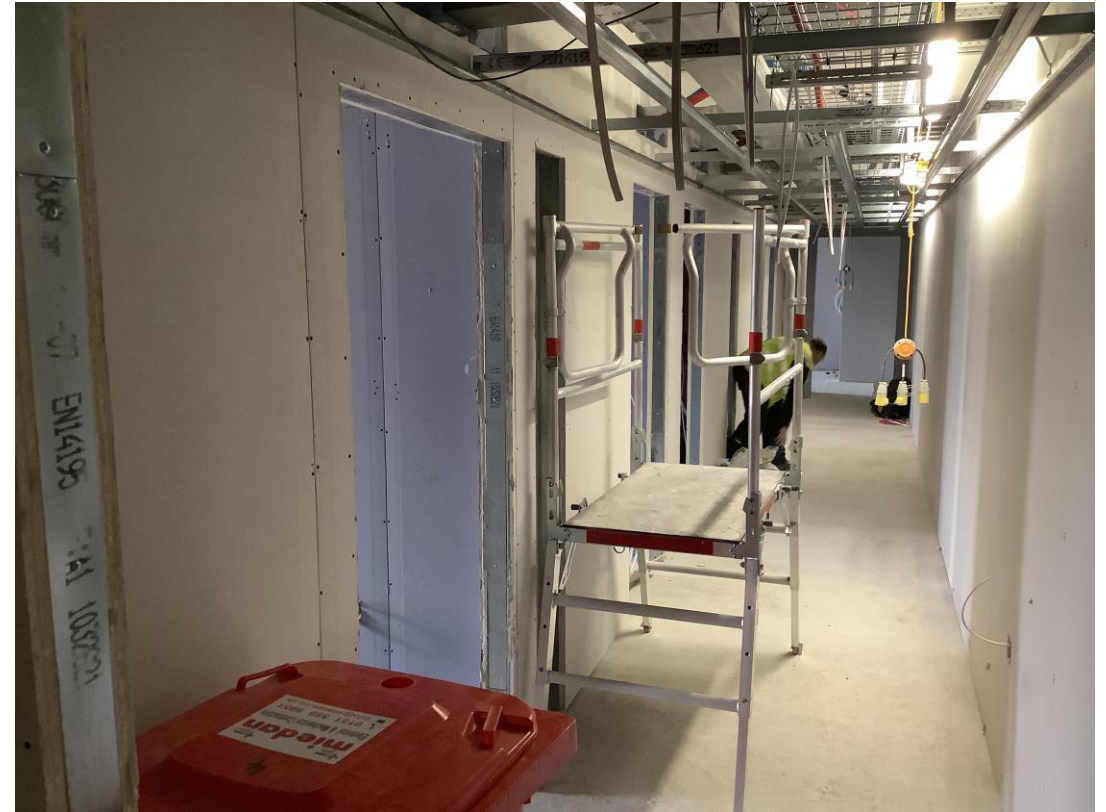
Student wing - Cluster rooms, general view
