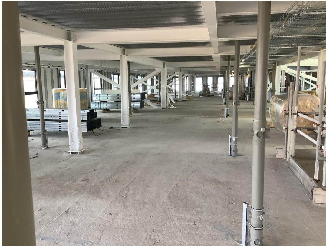
Residential wing - General progress to upper floor
