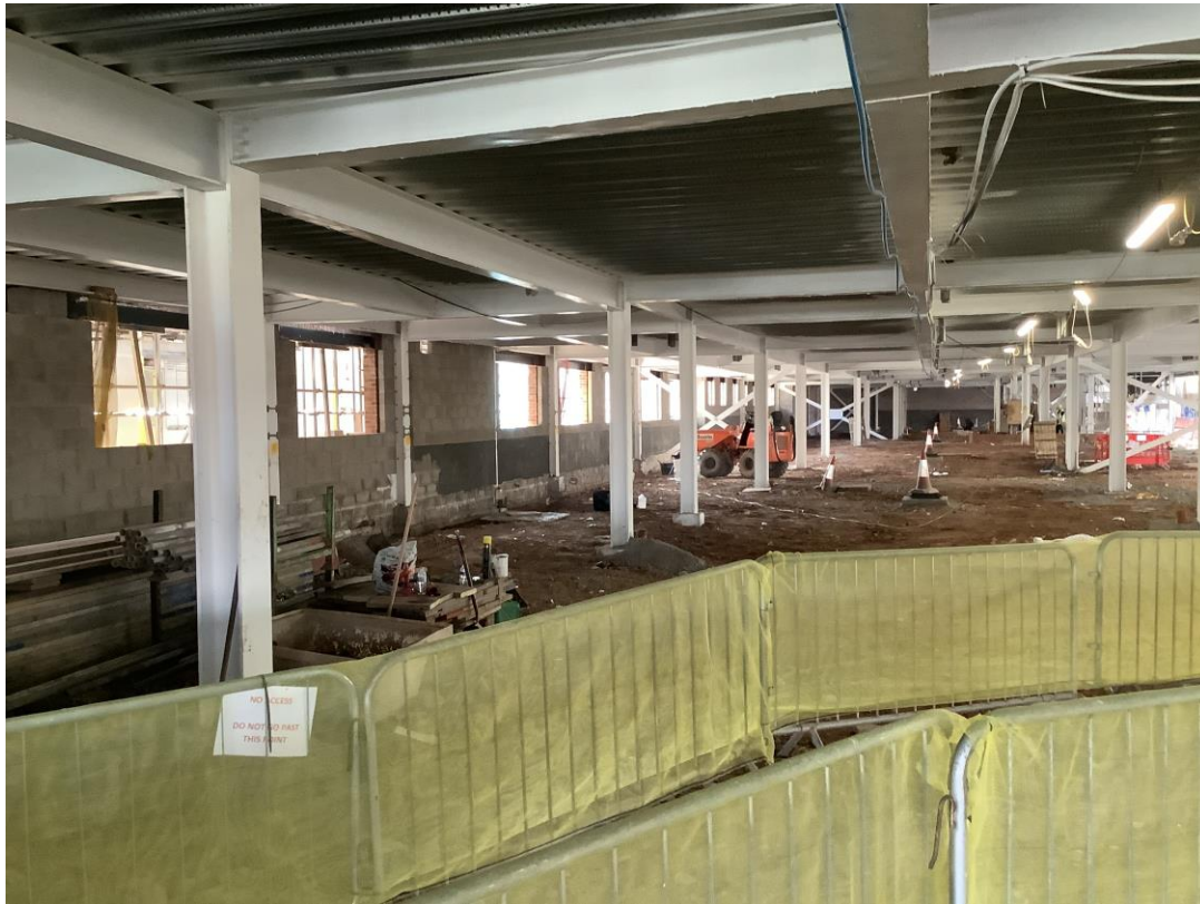
Ground floor - General progress photo
