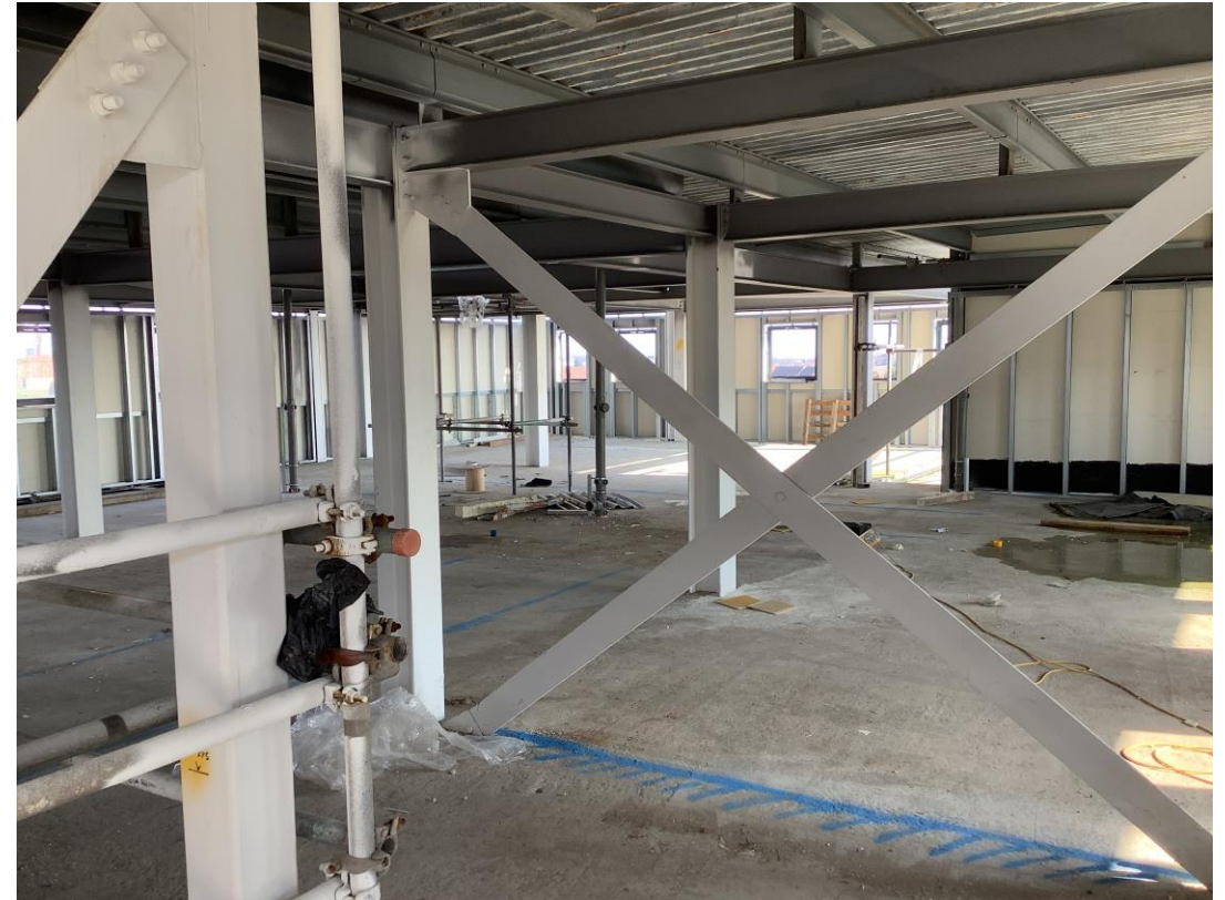
Student wing - General progress to upper floor
