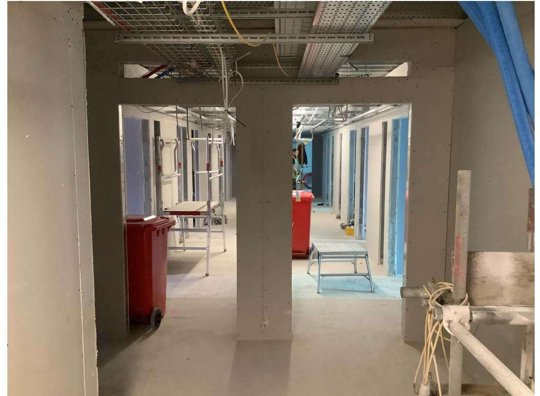
Student wing - Cluster rooms, general view
