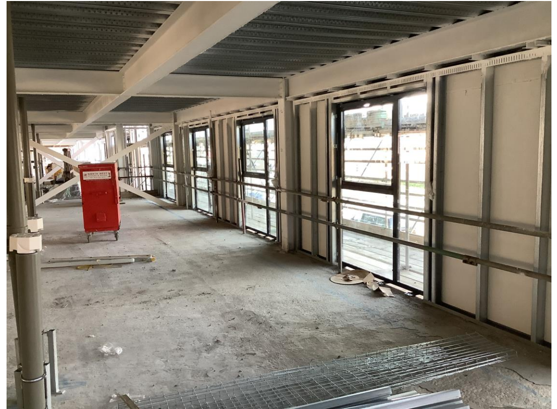
Residential wing - SFS & windows
