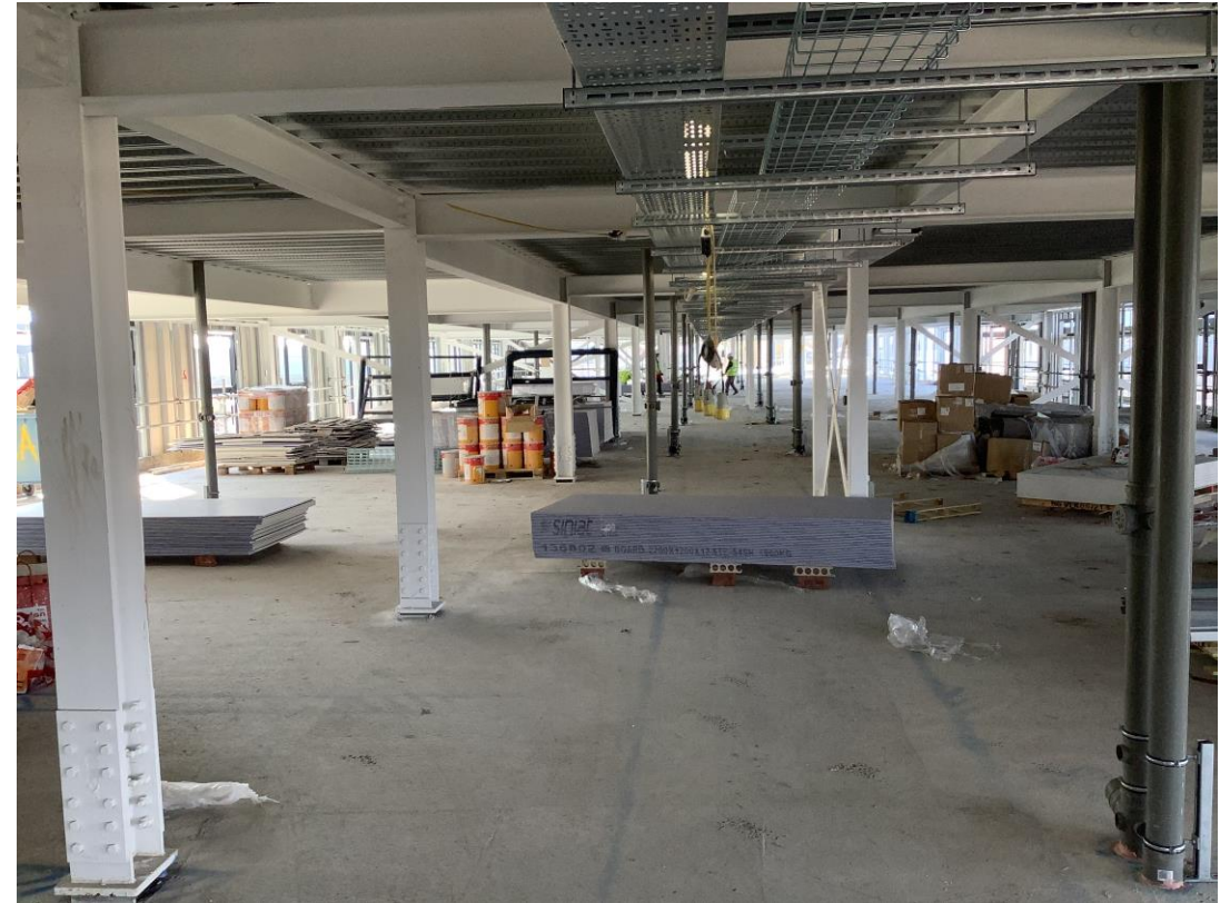
Residential wing - General progress to upper floor
