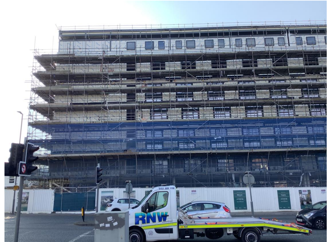
West Derby Road - Site view
