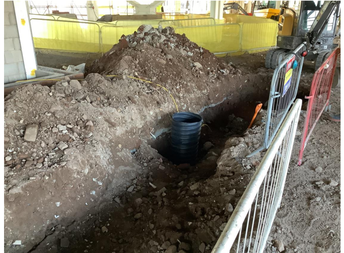
Ground floor trenching works for drainage
