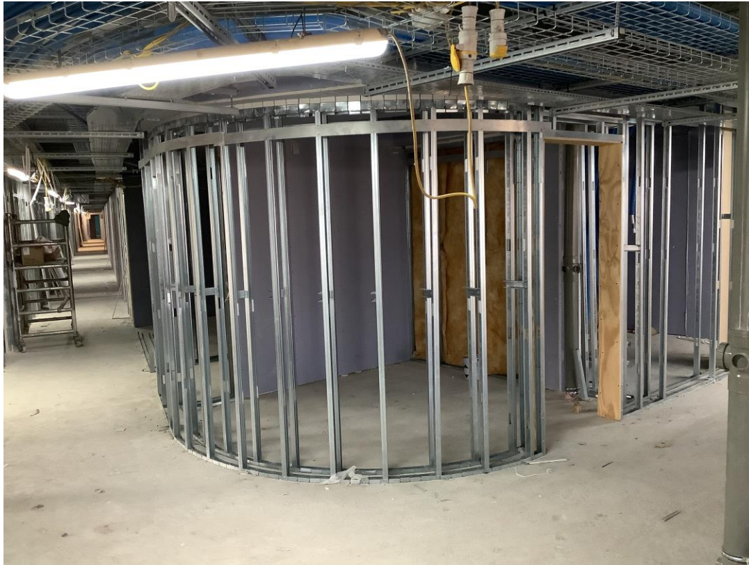
Student wing - Internal metal framework & plasterboard
