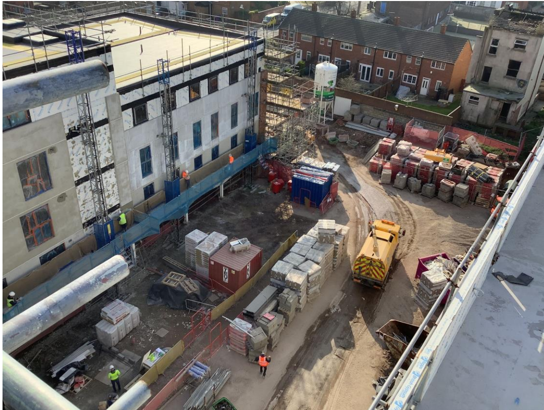
Inner courtyard - General site activity
