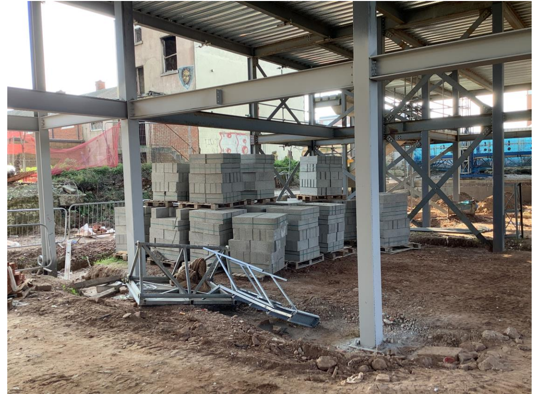
Commercial block - Intumescent coating progress
