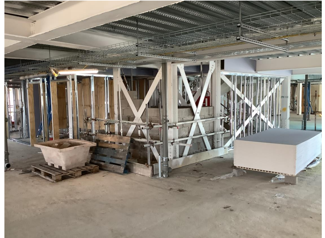
Student wing - Blockwork and metal framework to stair core
