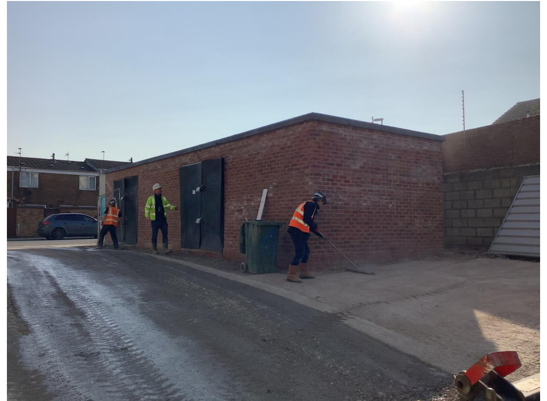
Brickwork and roof complete to sub-station
