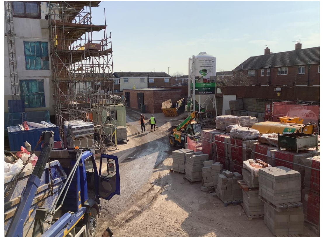
Commercial block view - General site activity
