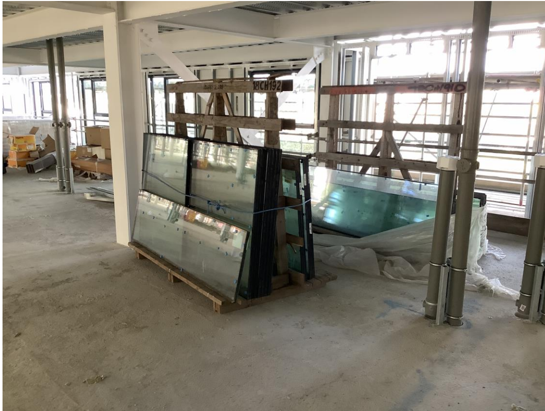
Material storage - Glazing units
