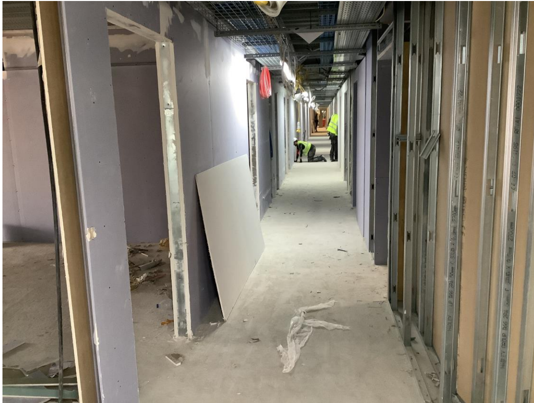
Student wing - Internal metal partitions & plasterboard
