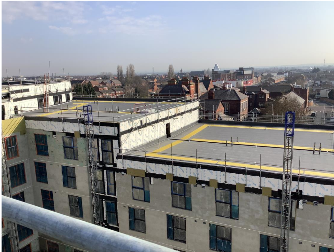
Student wing - Flat roof coverings, walkway matting & mansafe system
