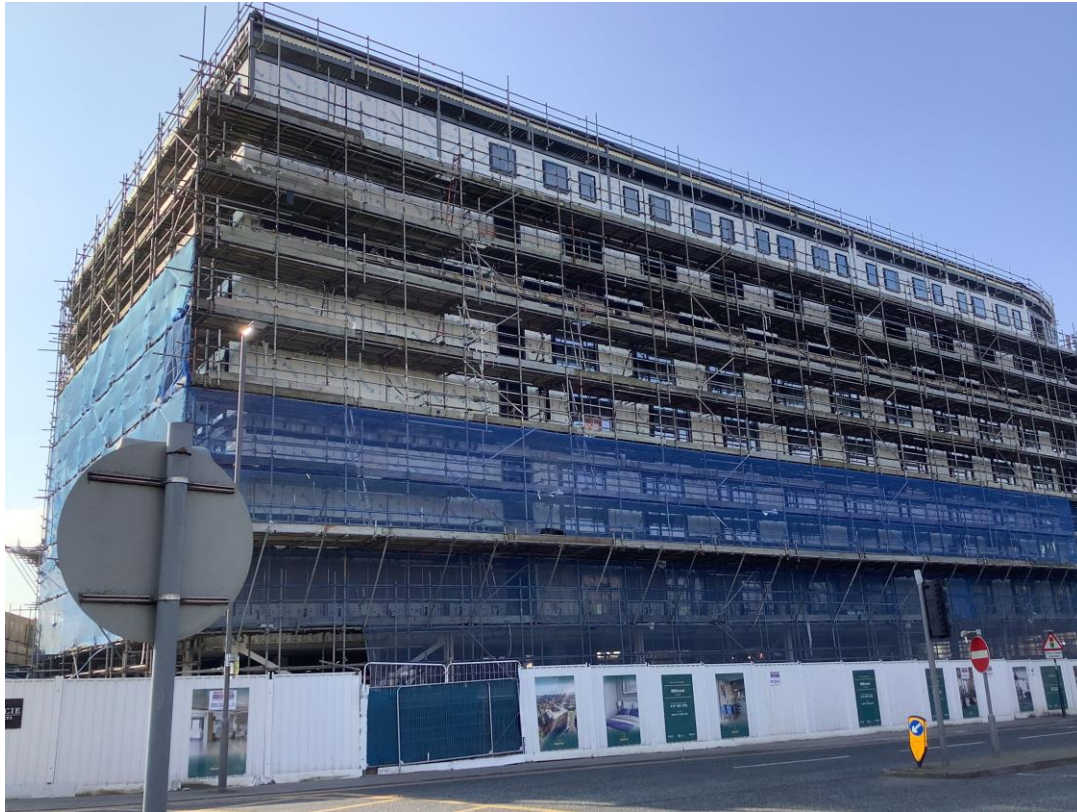
West Derby Road - Site view
