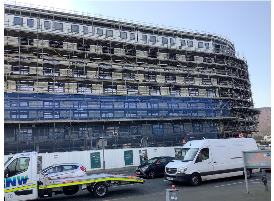
West Derby Road - Site view
