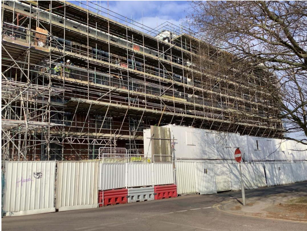
Walker Street - Site view
