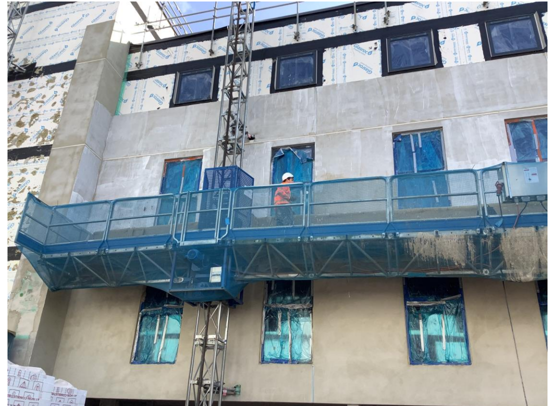
Student wing - Mast climbers, external insulation & render progress
