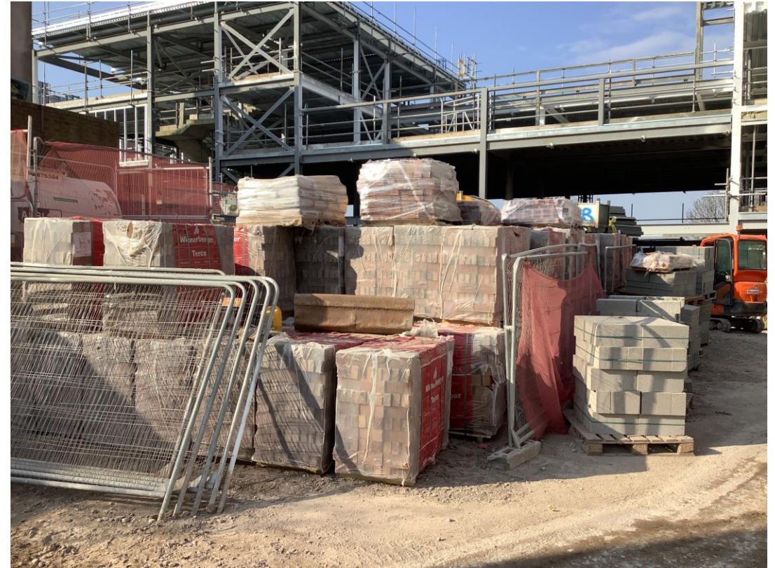
Material storage - Red brick and industrial blocks
