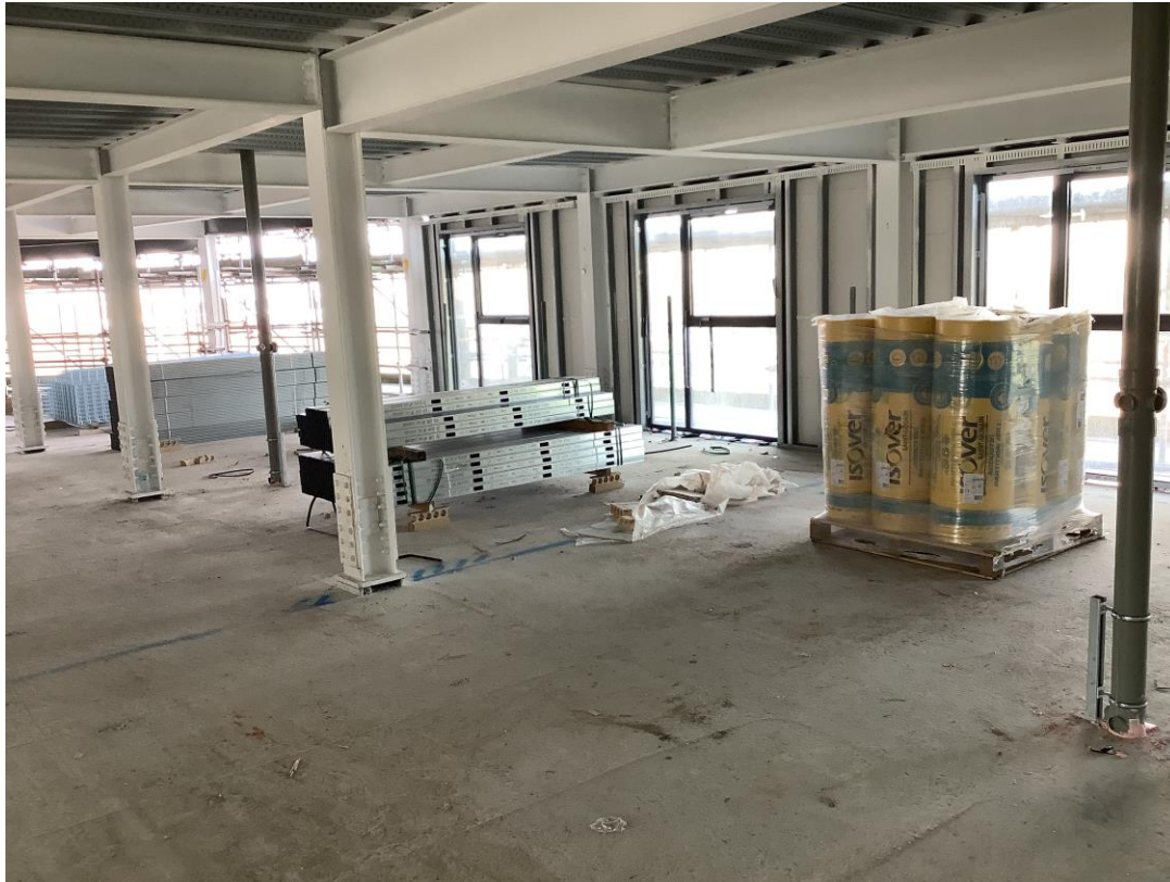
Material storage - Cable trays & internal insulation
