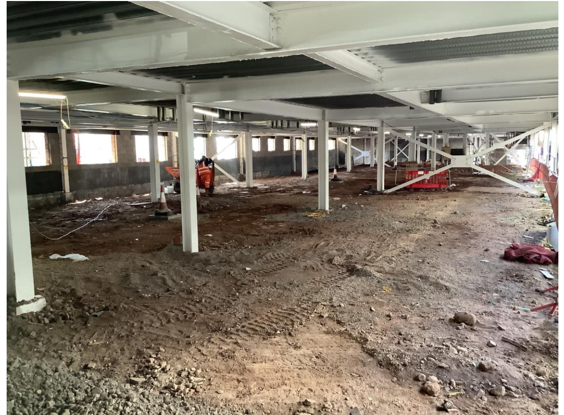
Ground floor - General progress photo
