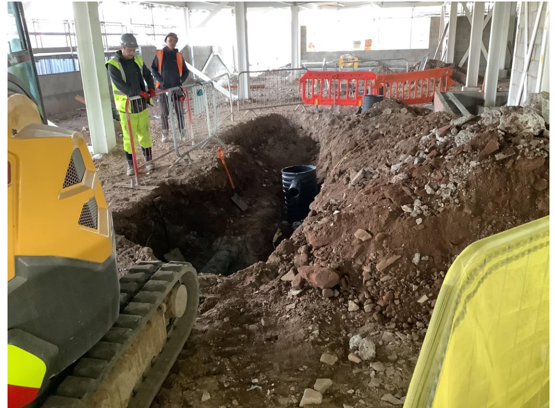
Under ground drainage
