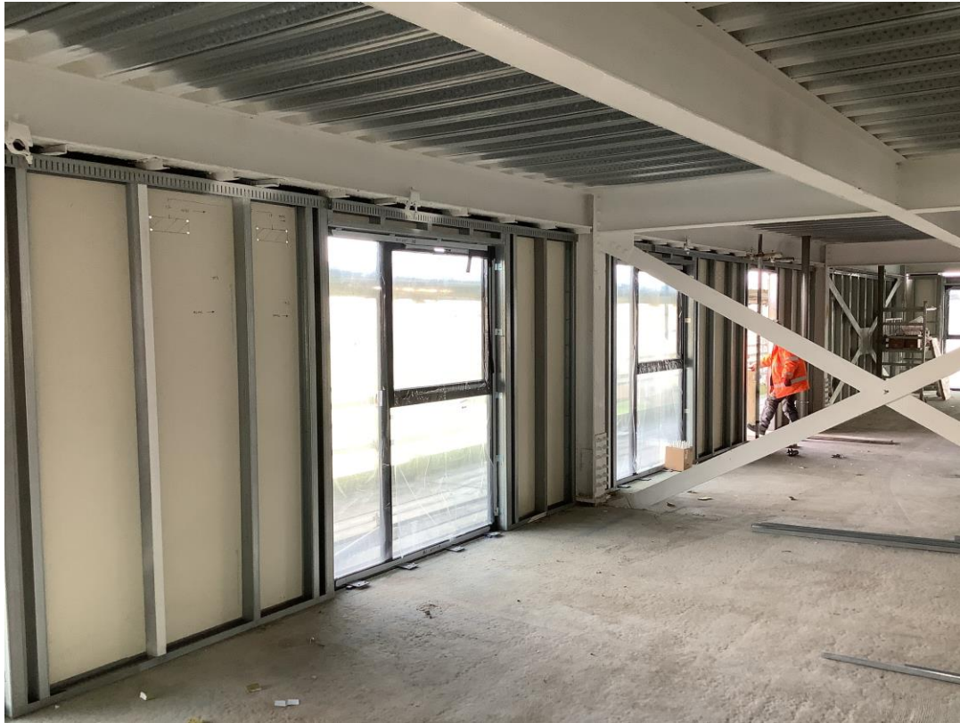
Residential wing - Windows
