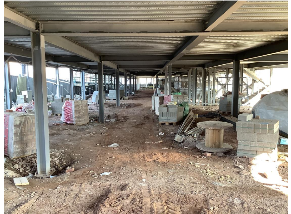
Commercial block - General progress photo
