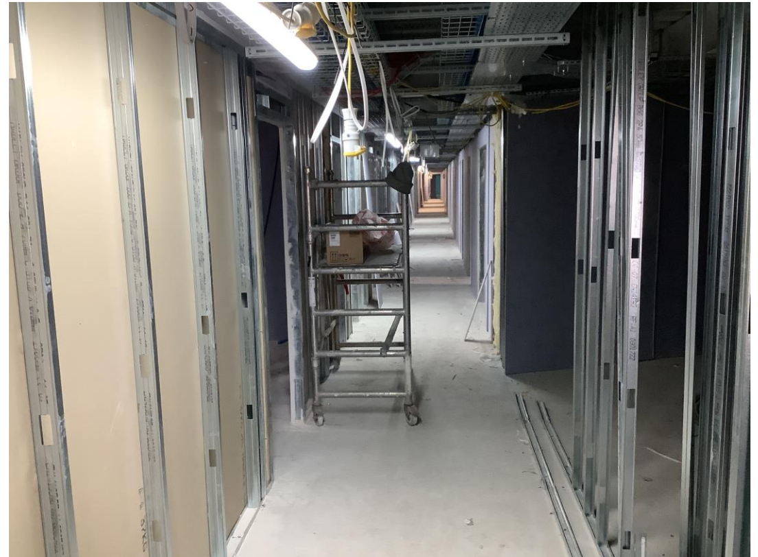
Student wing - Internal metal partitions & plasterboard progress
