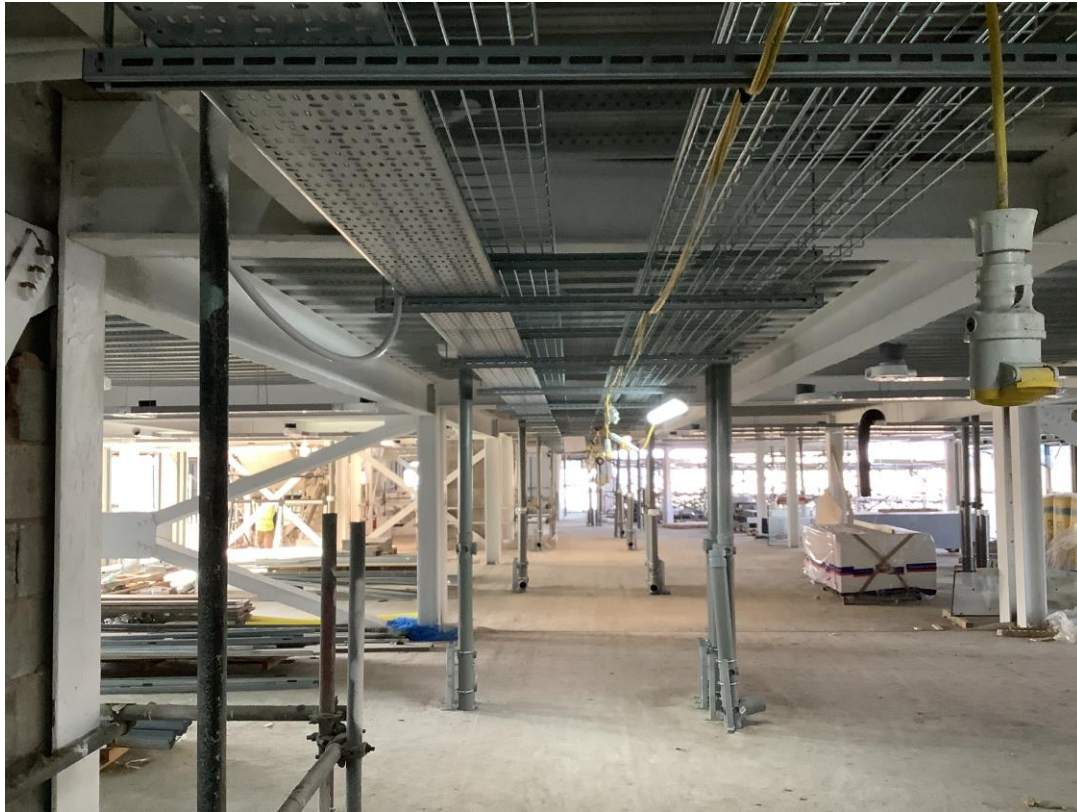
Residential wing - General progress photo
