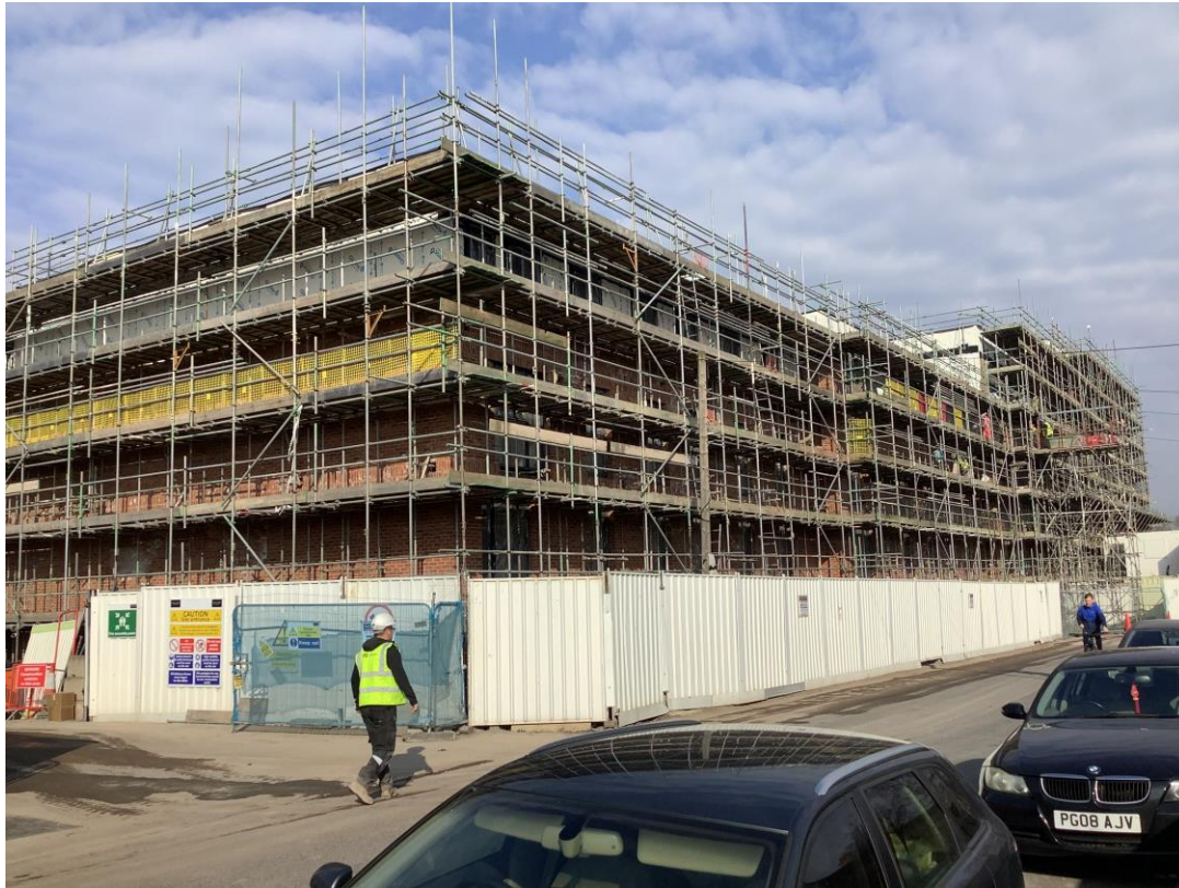
Walker Street - Site view
