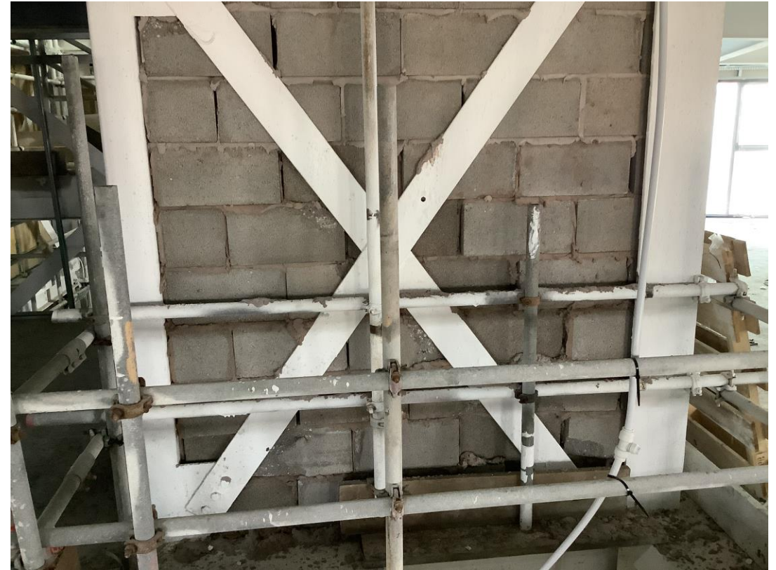
Student wing - Blockwork to stair core
