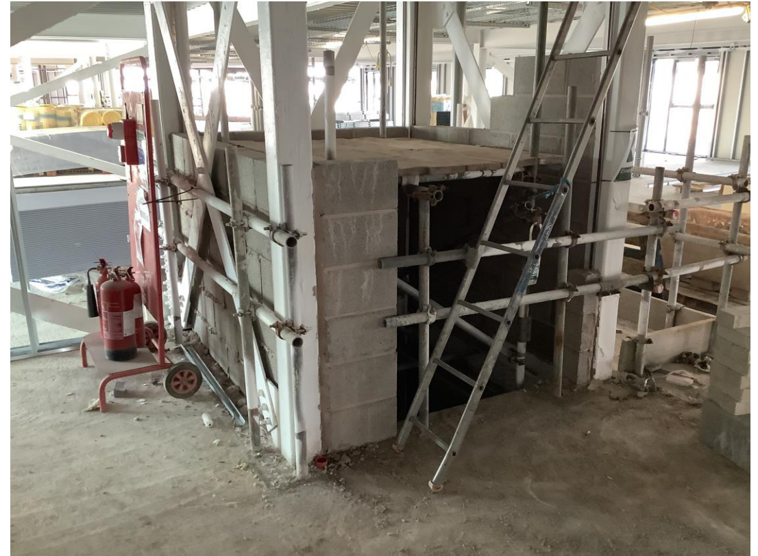
Student wing - Blockwork to stair core
