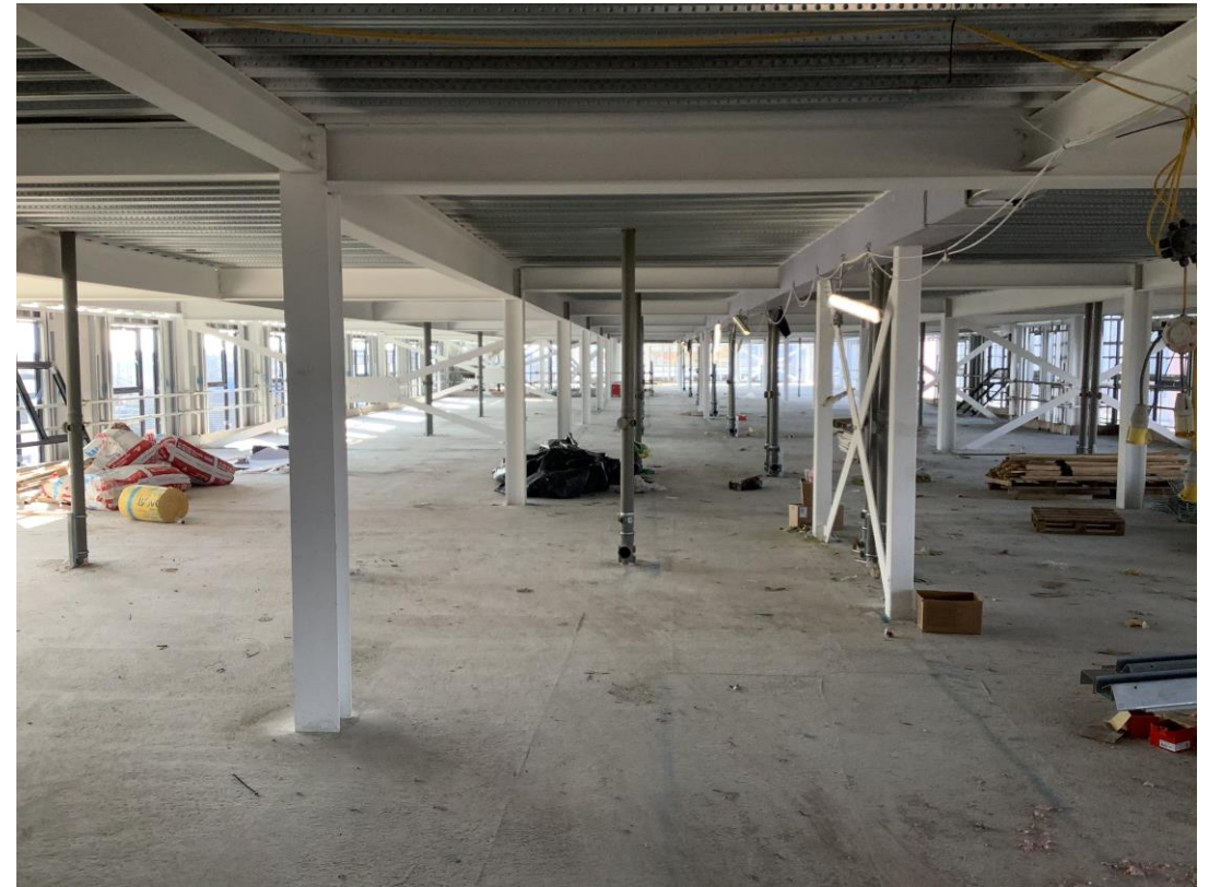
Residential wing - First fix Mechanical works
