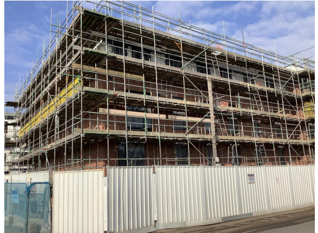
Walker Street - Site view
