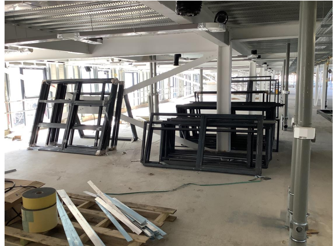
Material storage - Window frames
