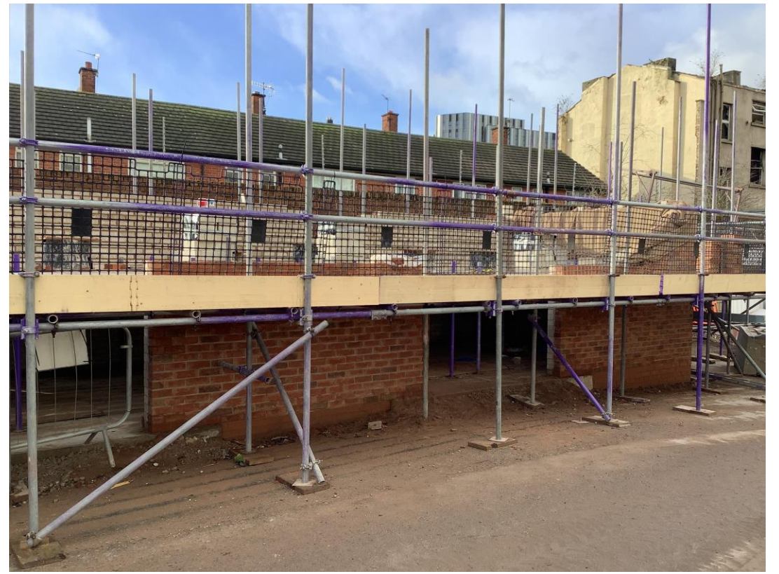
Brickwork progress to sub-station
