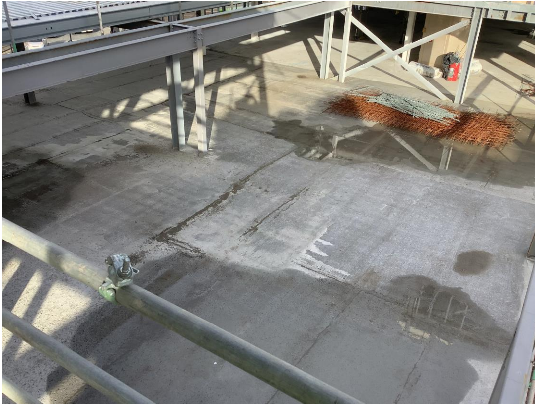
Commercial block - Concrete floor slab
