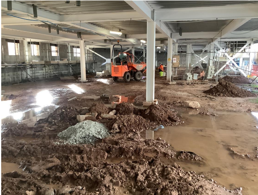
Student wing - Ground floor slab preparations
