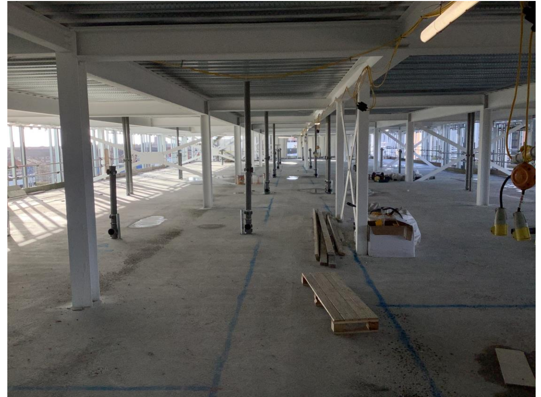
Residential wing - Setting out partitions
