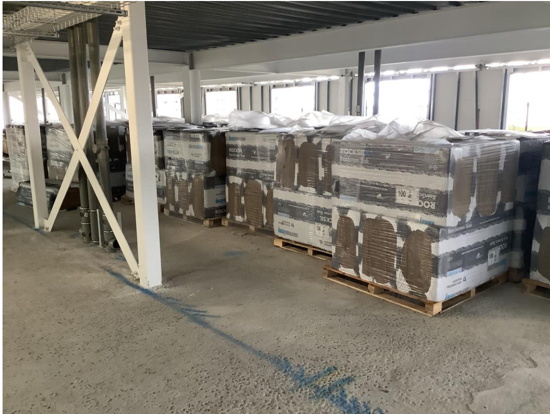
Material storage - Insulation
