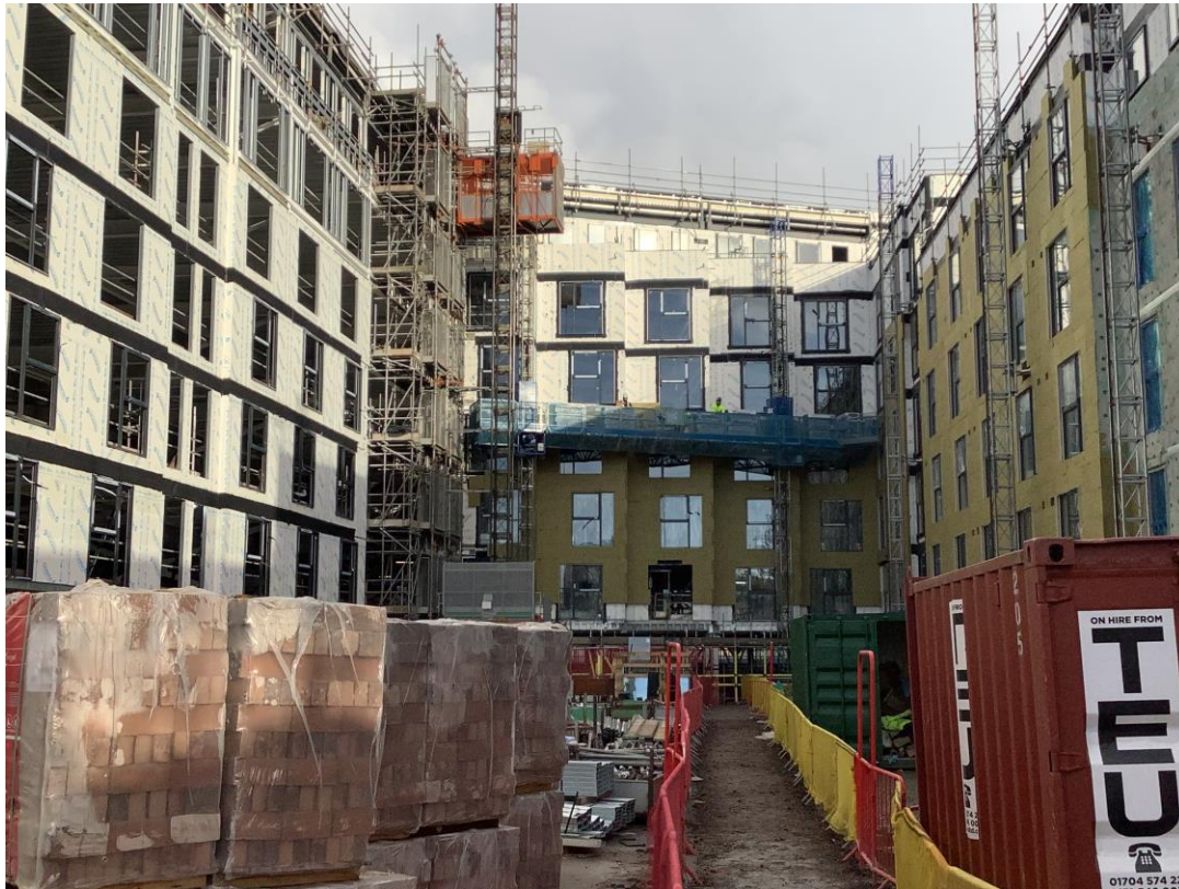
Inner courtyard - General site view
