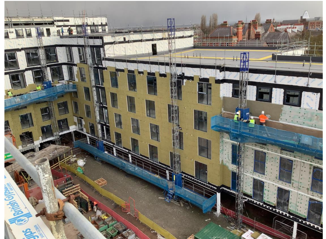
Student wing - External insulation & render progress
