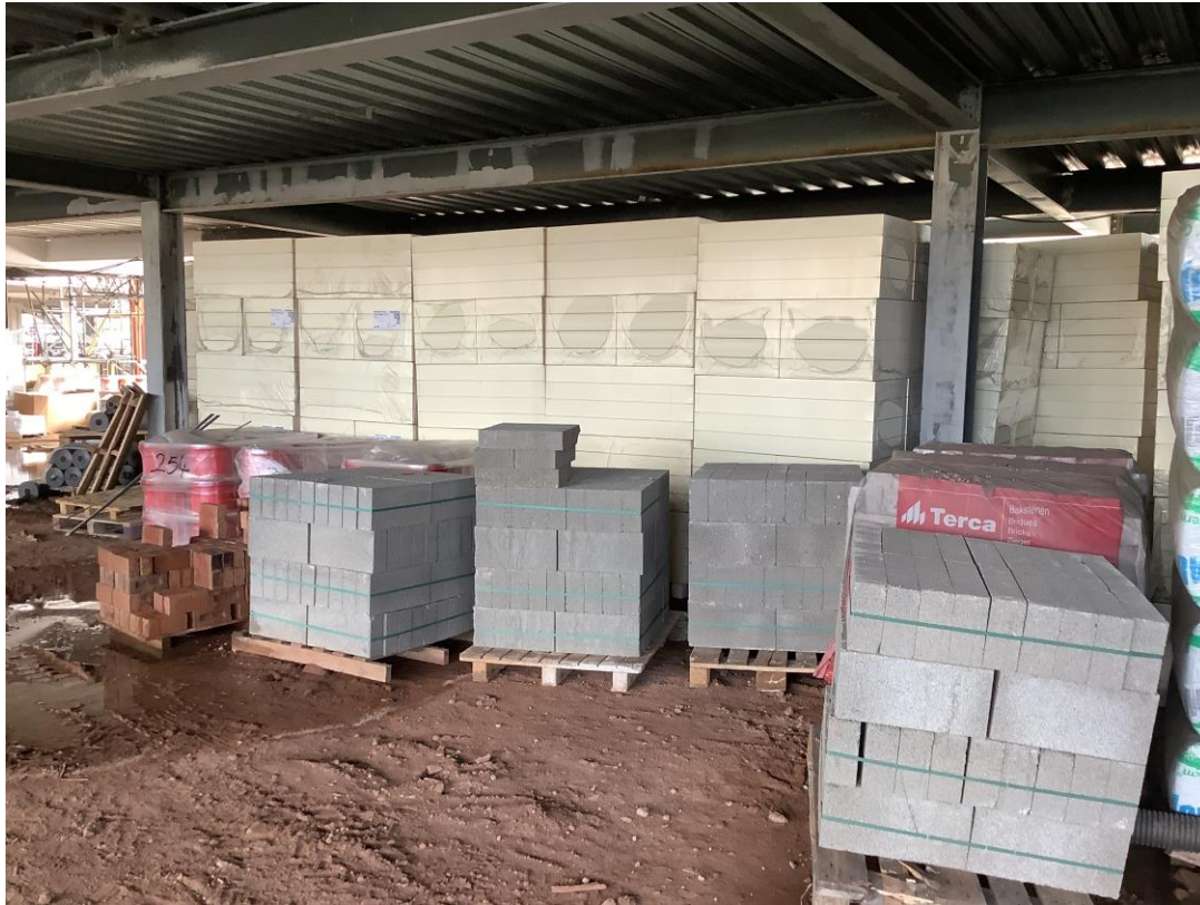
Material storage - Industrial block and insulation
