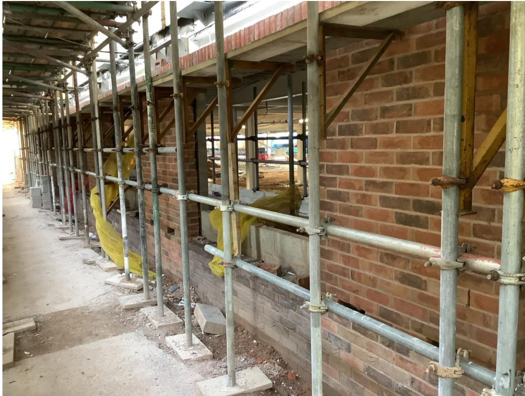
Student wing - External facing brick ongoing
