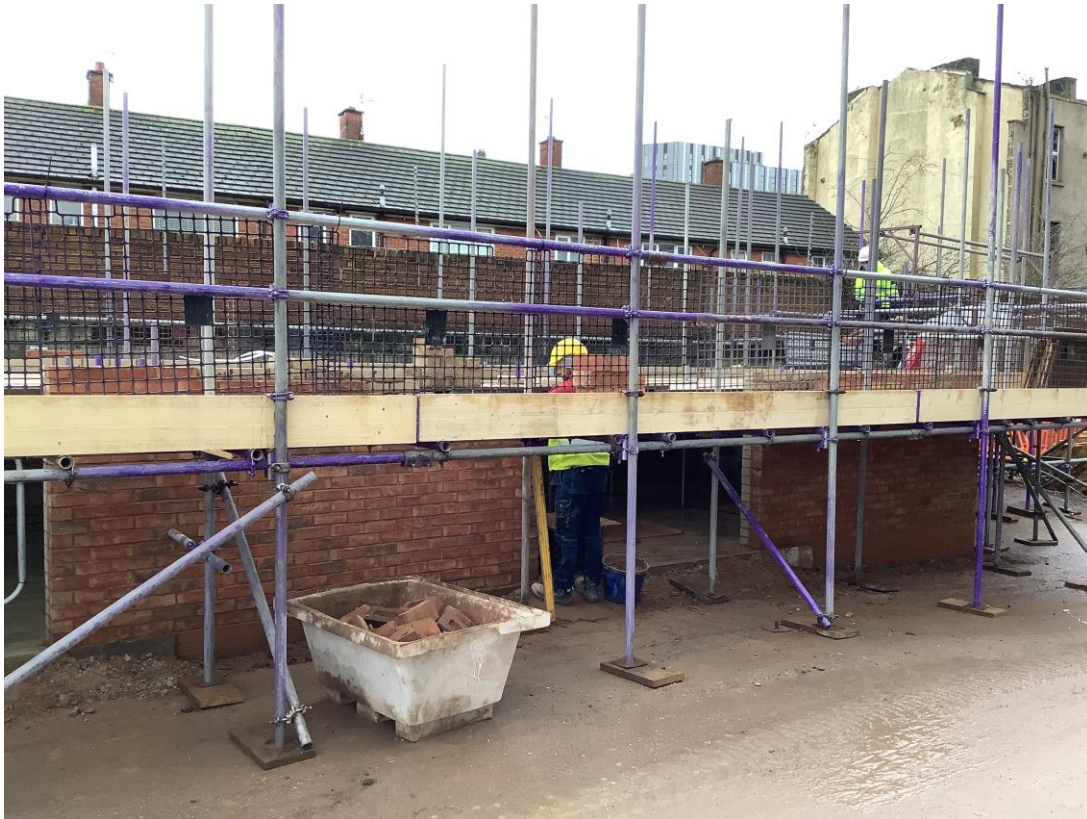
Brickwork progress to sub-station
