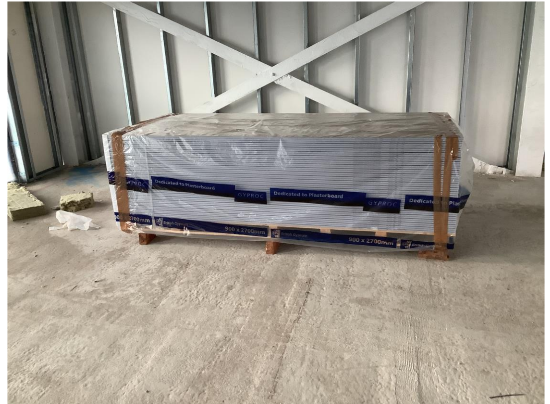
Material storage - Plasterboard
