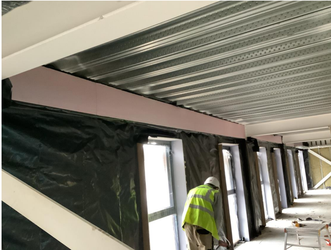
Student wing - Internal dry lining
