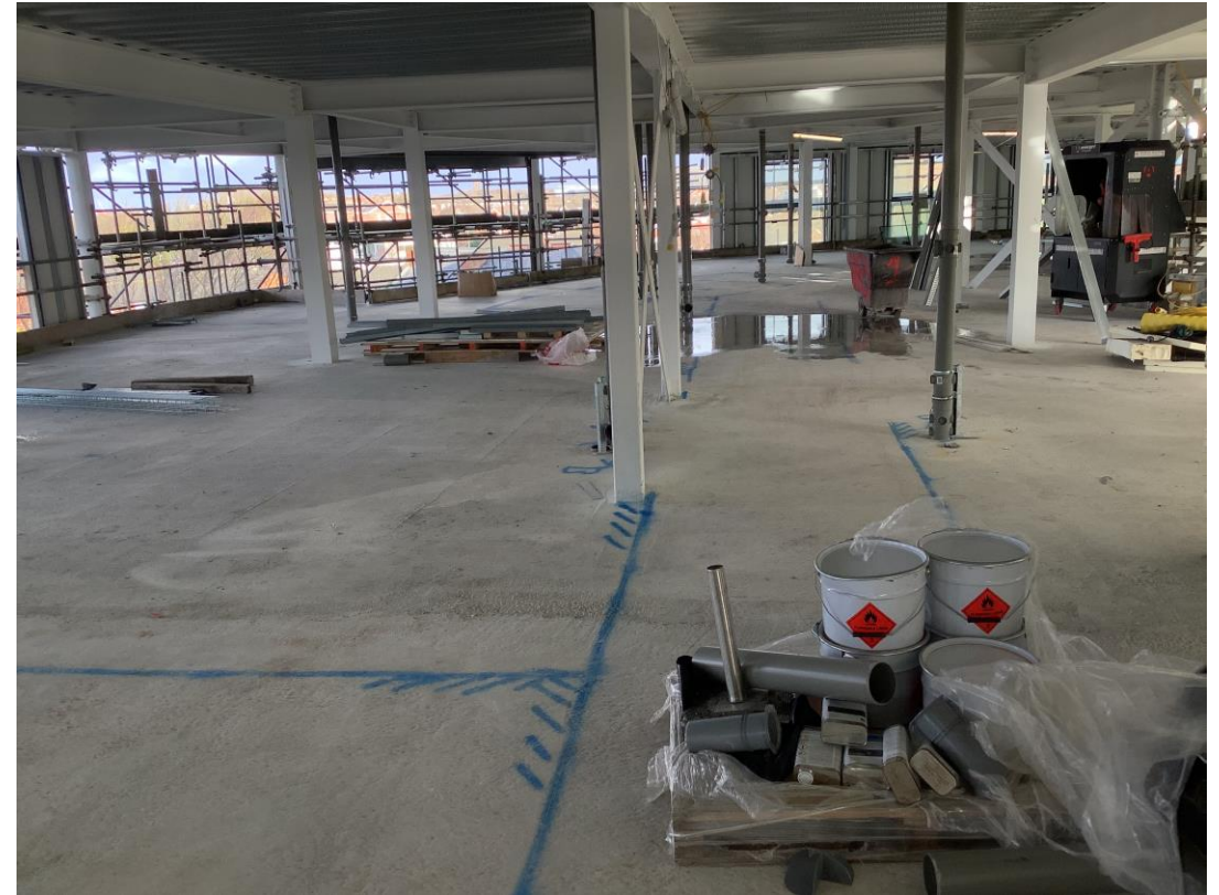
Residential wing - Setting out partitions
