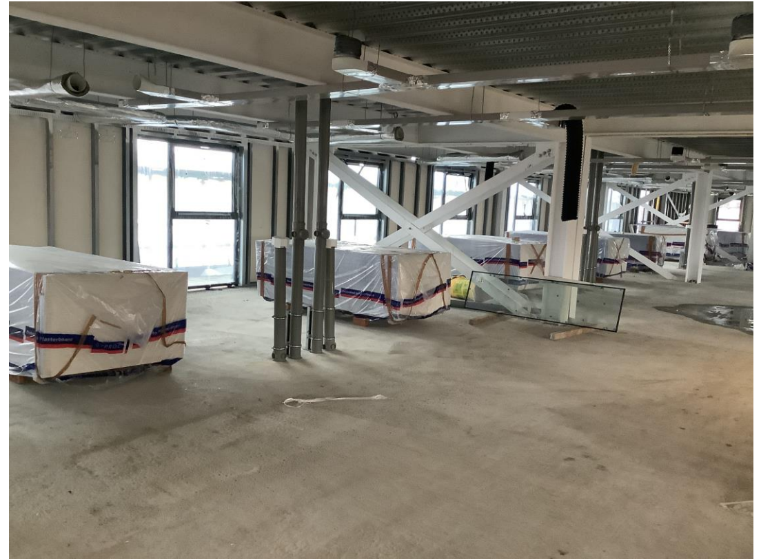
Material storage - Plasterboard
