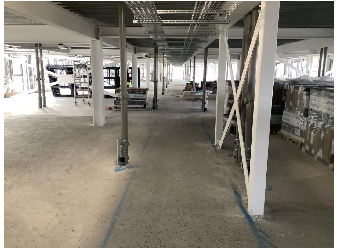
Residential wing - First fix Mechanical works and setting out partitions
