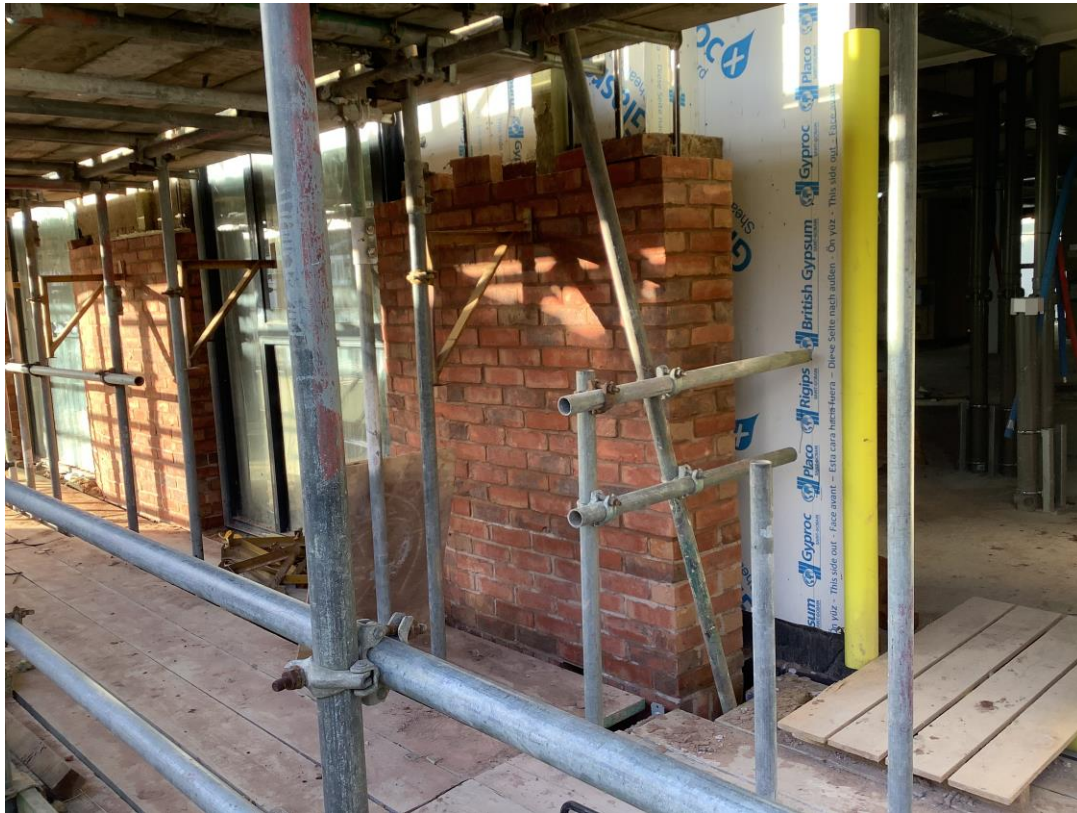
Student wing - External facing brick ongoing
