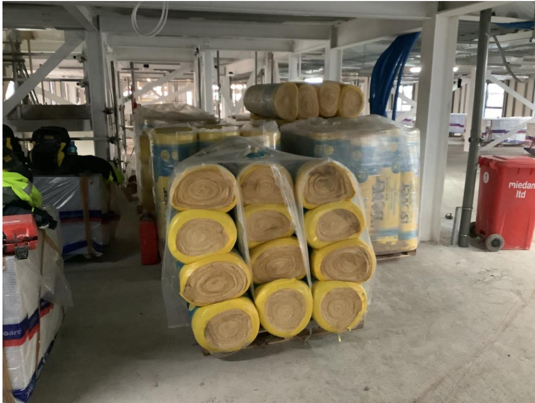
Material storage - Insulation
