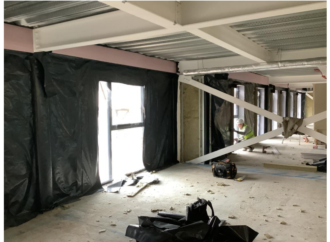
Student wing - Internal dry lining
