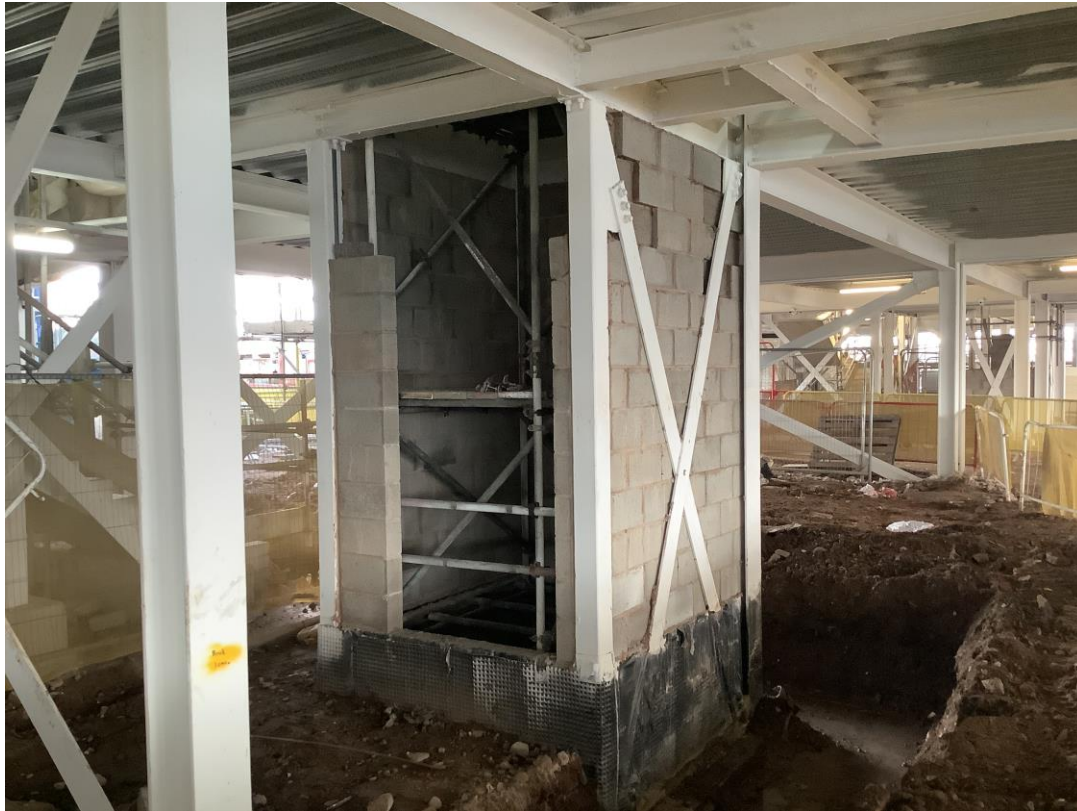
Student wing - Blockwork to stair cores
