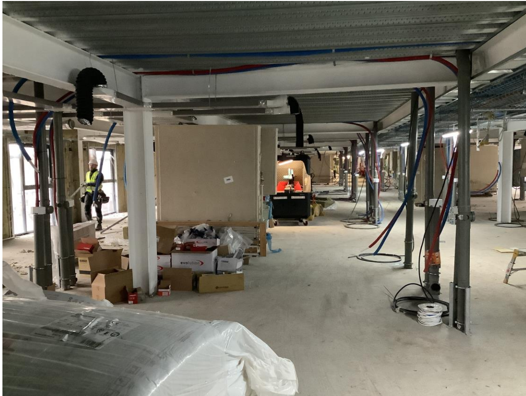
Student wing - First fix Mechanical & Electrical works
