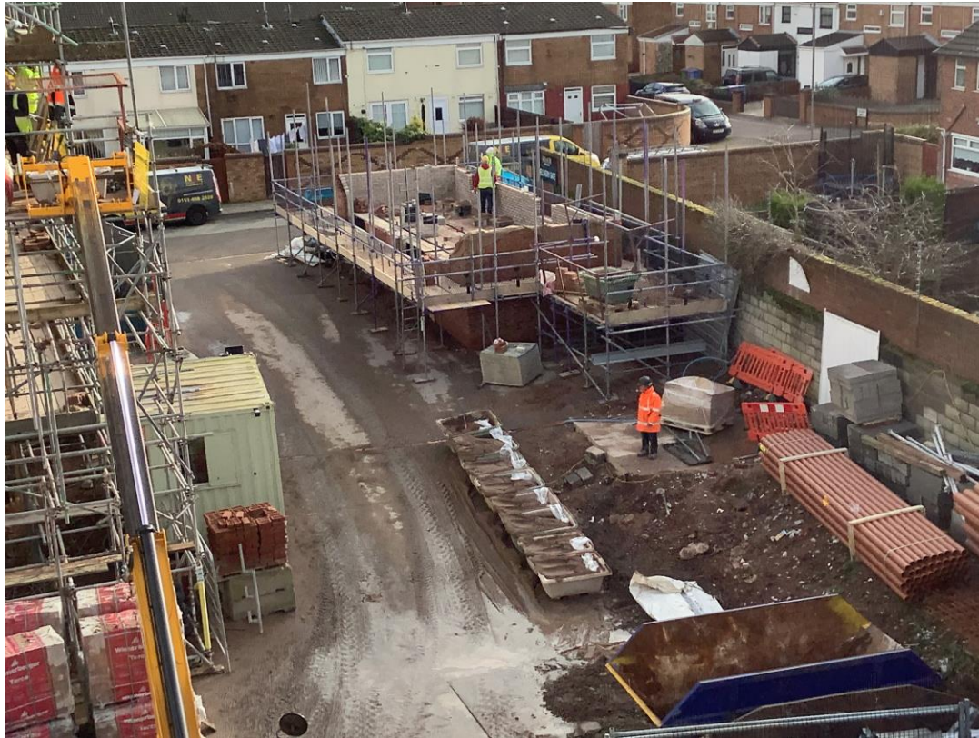
Residential wing view - Brickwork progress to sub-station
