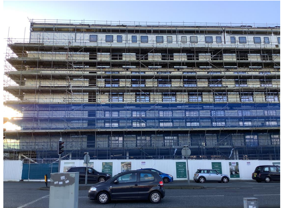
West Derby Road - Site view
