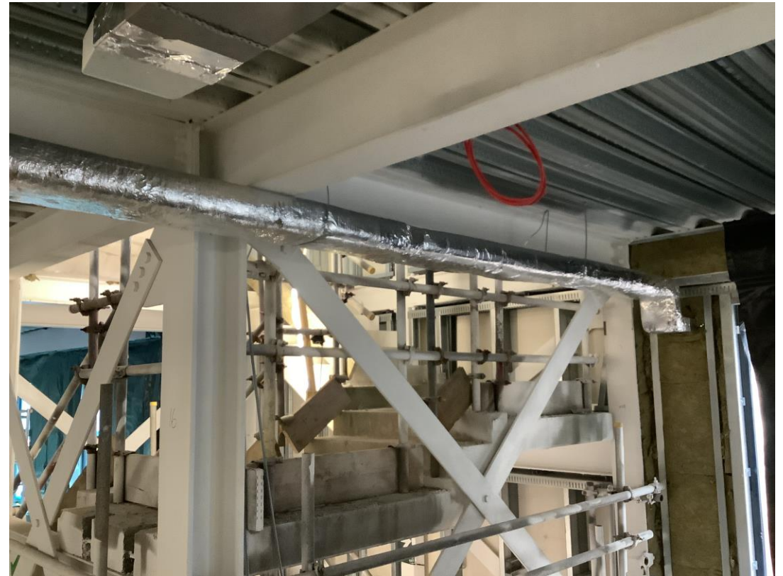
Student wing - First fix Mechanical works
