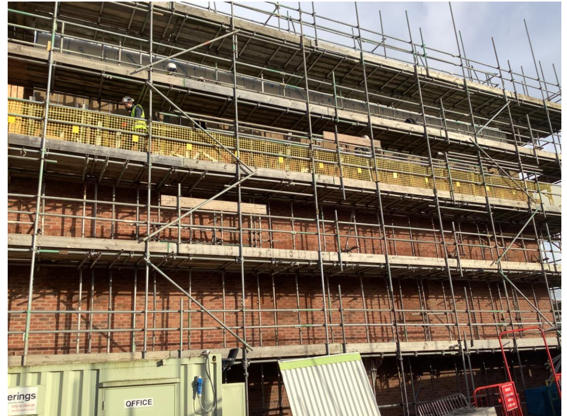
Student wing - Gable end facing brick ongoing
