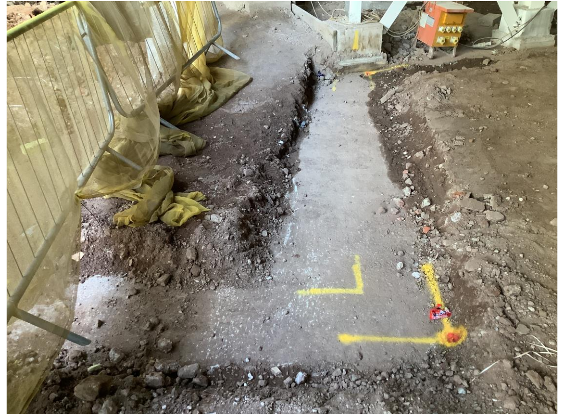
Student wing - Ground floor slab preparations
