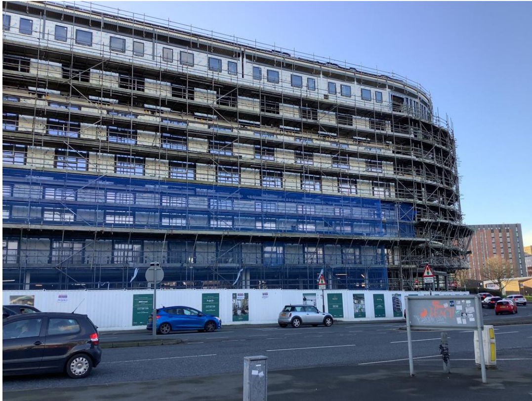
West Derby Road - Site view
