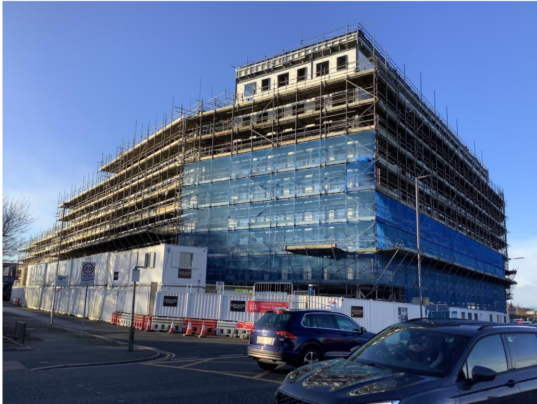
West Derby Road - Site view
