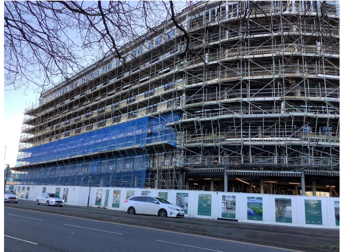
West Derby Road - Site view
