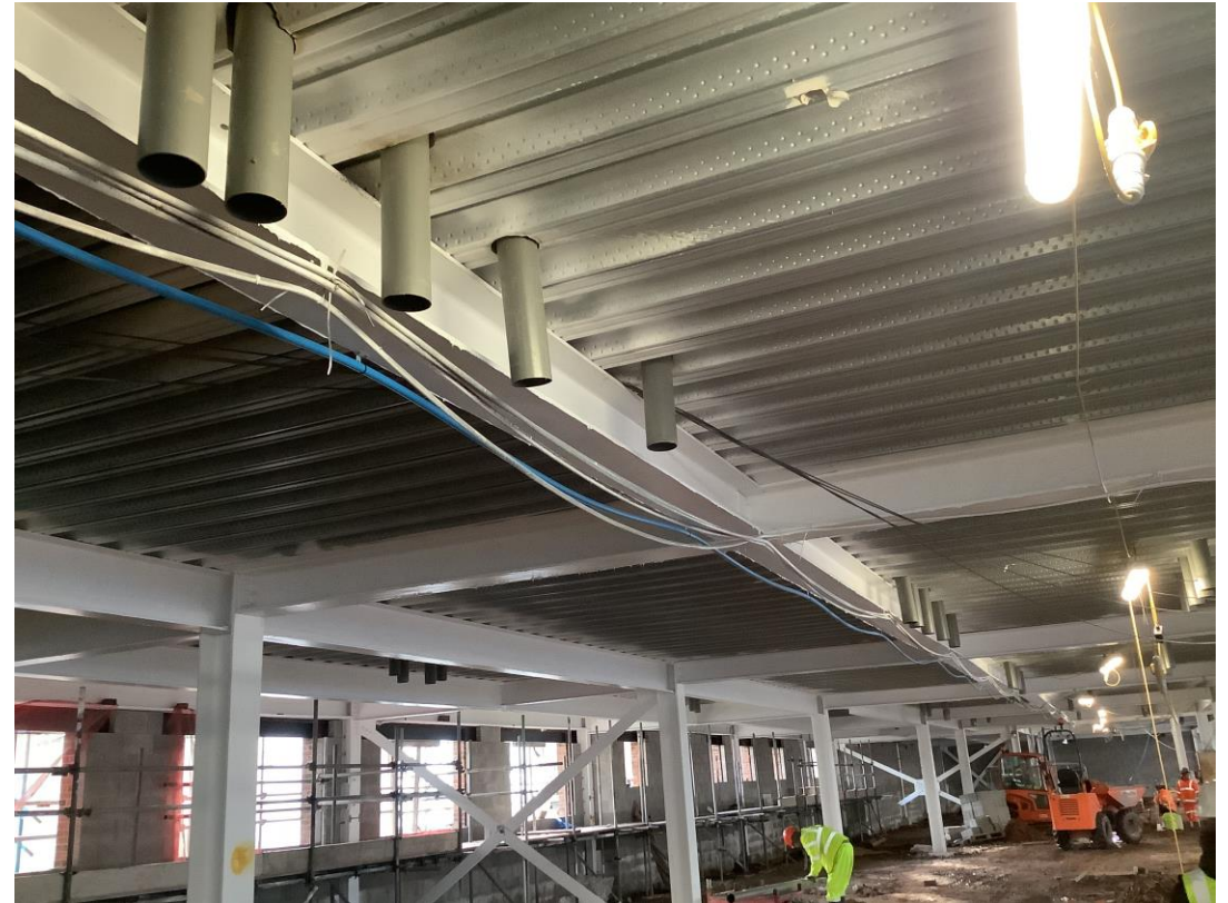
Student wing - First fix Mechanical works
