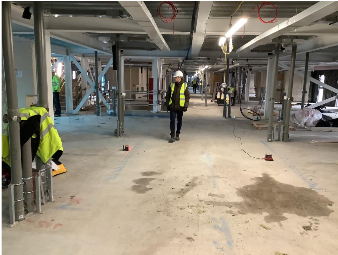
Student wing - First fix Mechanical & Electrical works
