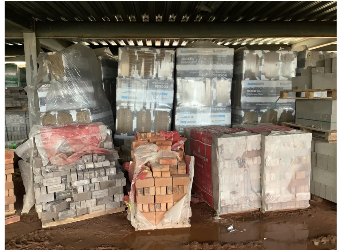
Material storage - Brick and insulation
