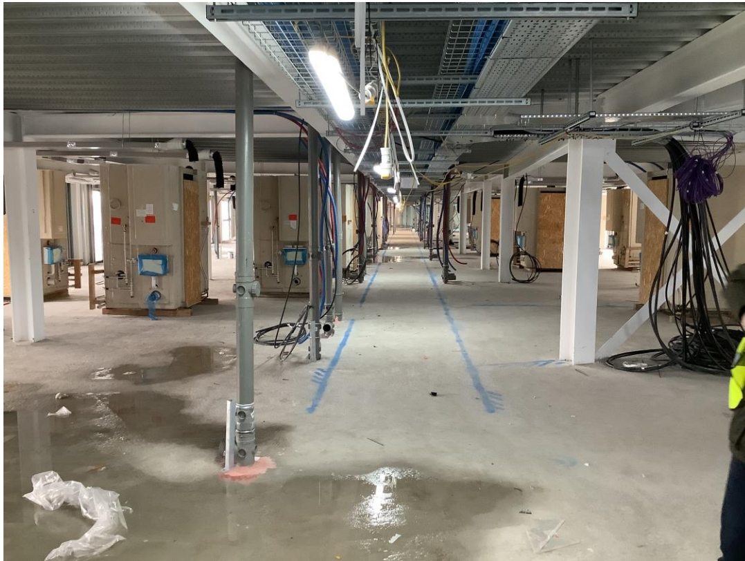
Student wing - First fix Mechanical & Electrical works and setting out partitions
