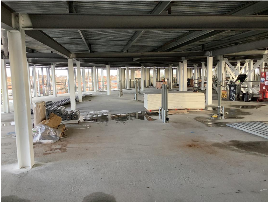
Student wing - General progress to upper floor
