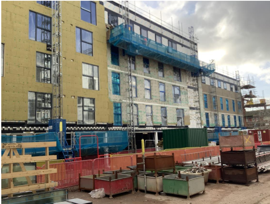
Student wing - External insulation & render progress
