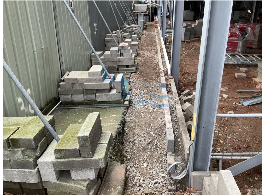
Commercial block - Retaining wall blockwork and back fill
