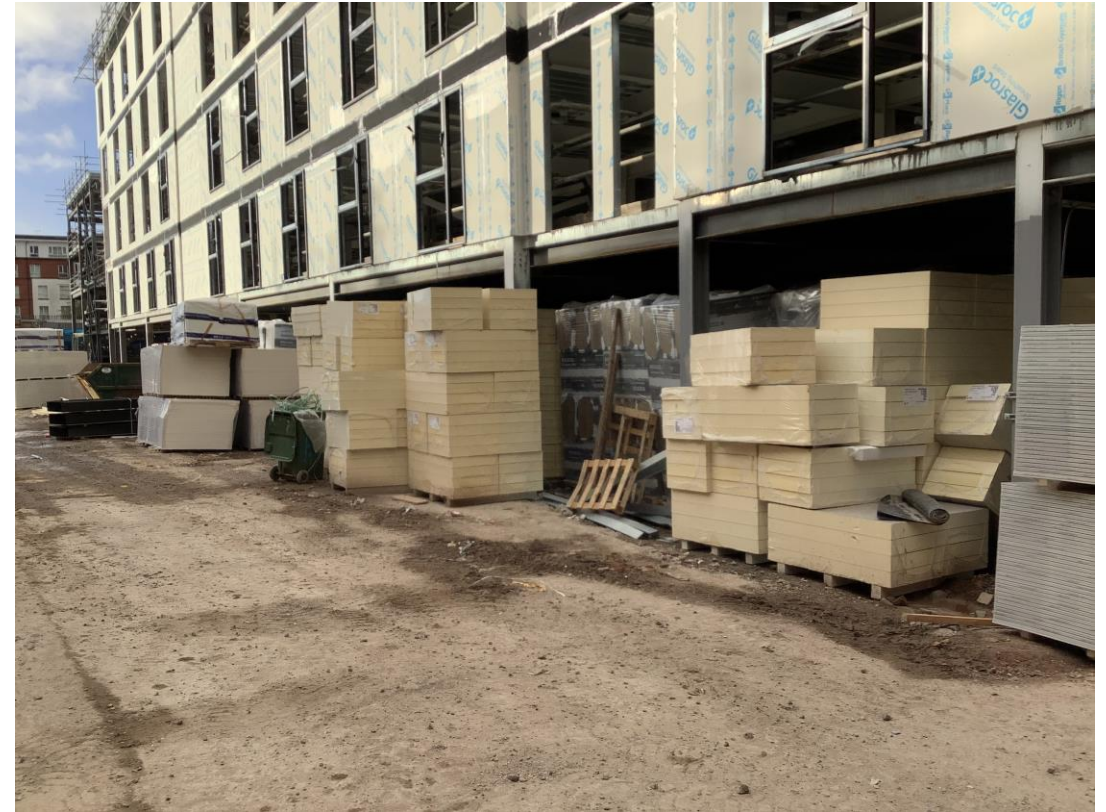
Material storage - Insulation
