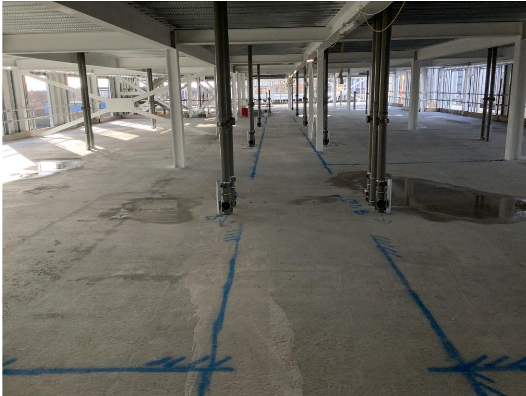
Residential wing - Setting out partitions
