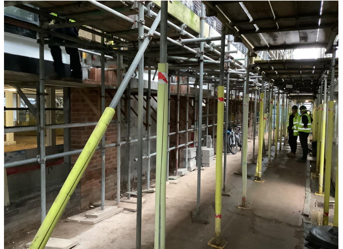
Student wing - External facing brick ongoing
