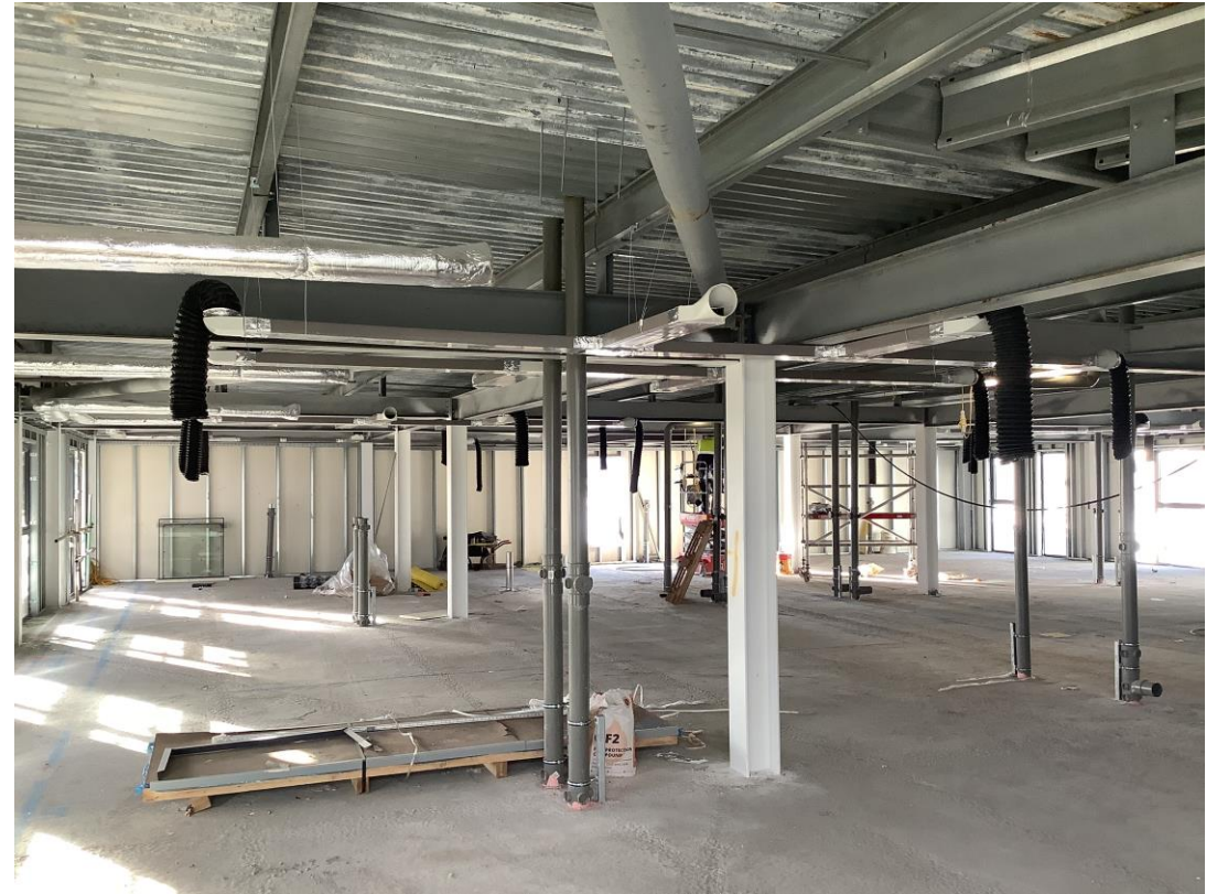
Student wing - First fix Mechanical works
