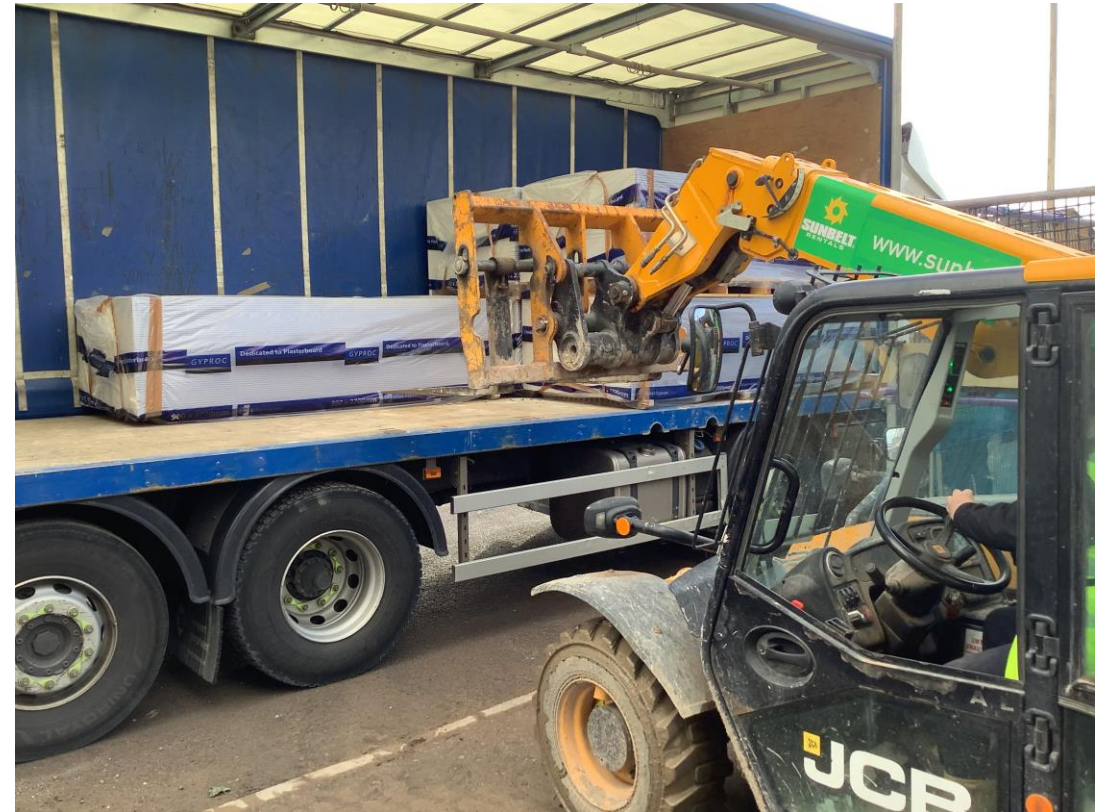
Materials delivery - Plasterboard
