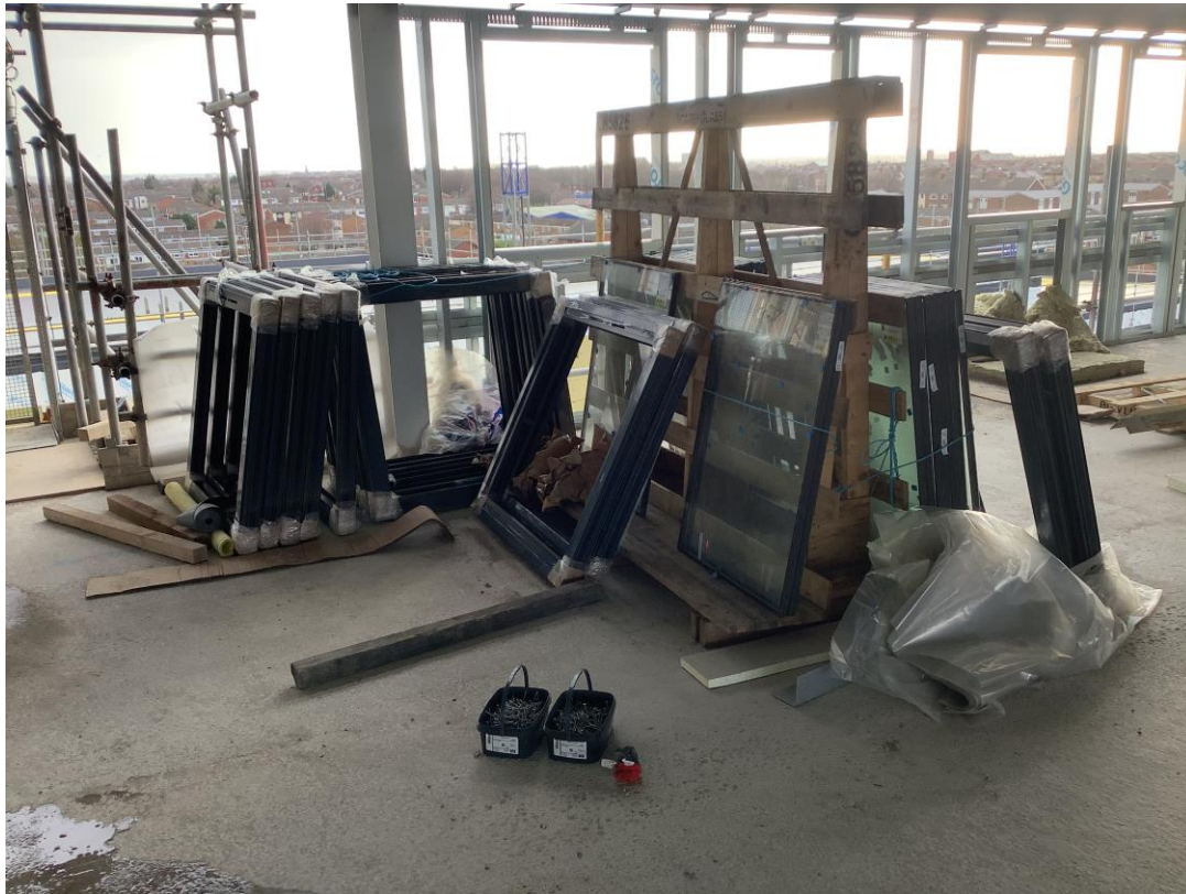
Material storage - Window frames and glazing units
