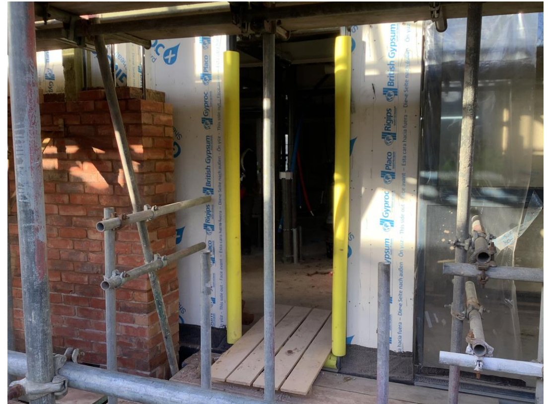
Student wing - External access on to scaffolding
