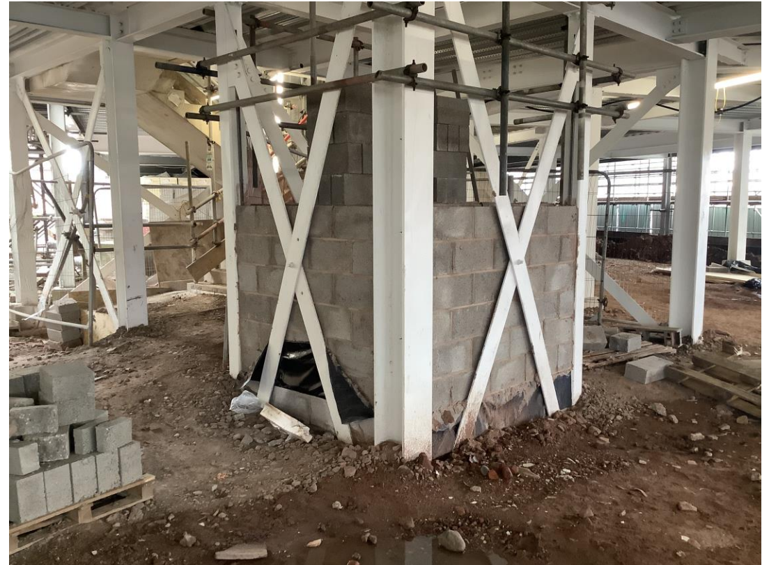
Student wing - Blockwork to stair cores
