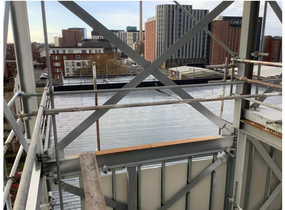
Commercial block - Flat roof structure
