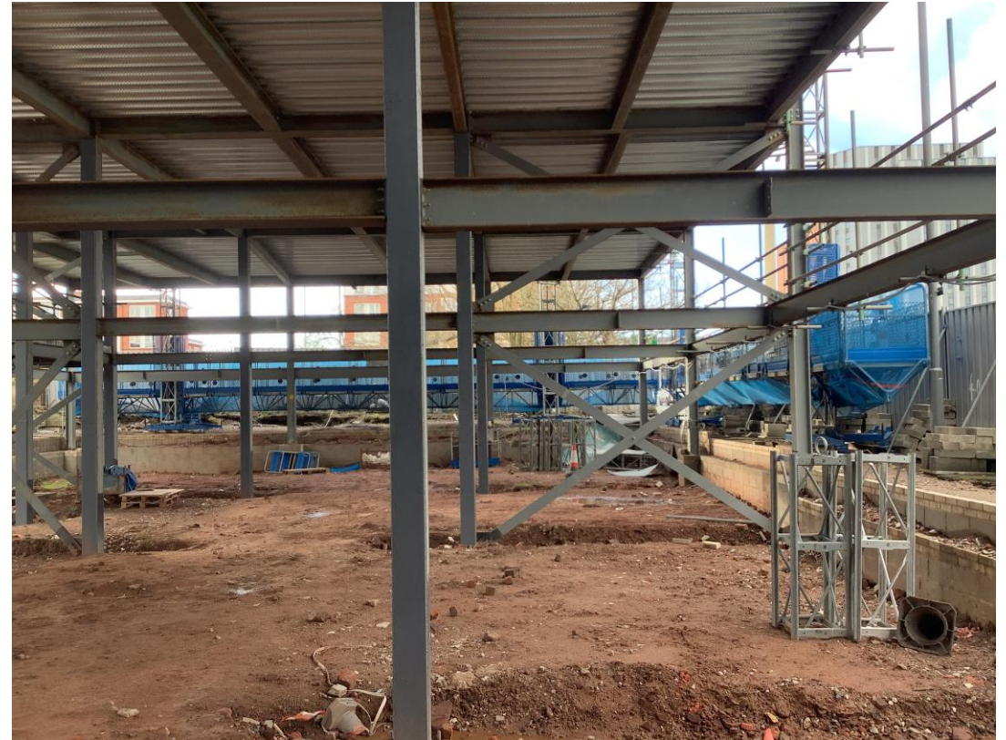
Commercial block - Metal frame structure, mast climbers and retaining wall
