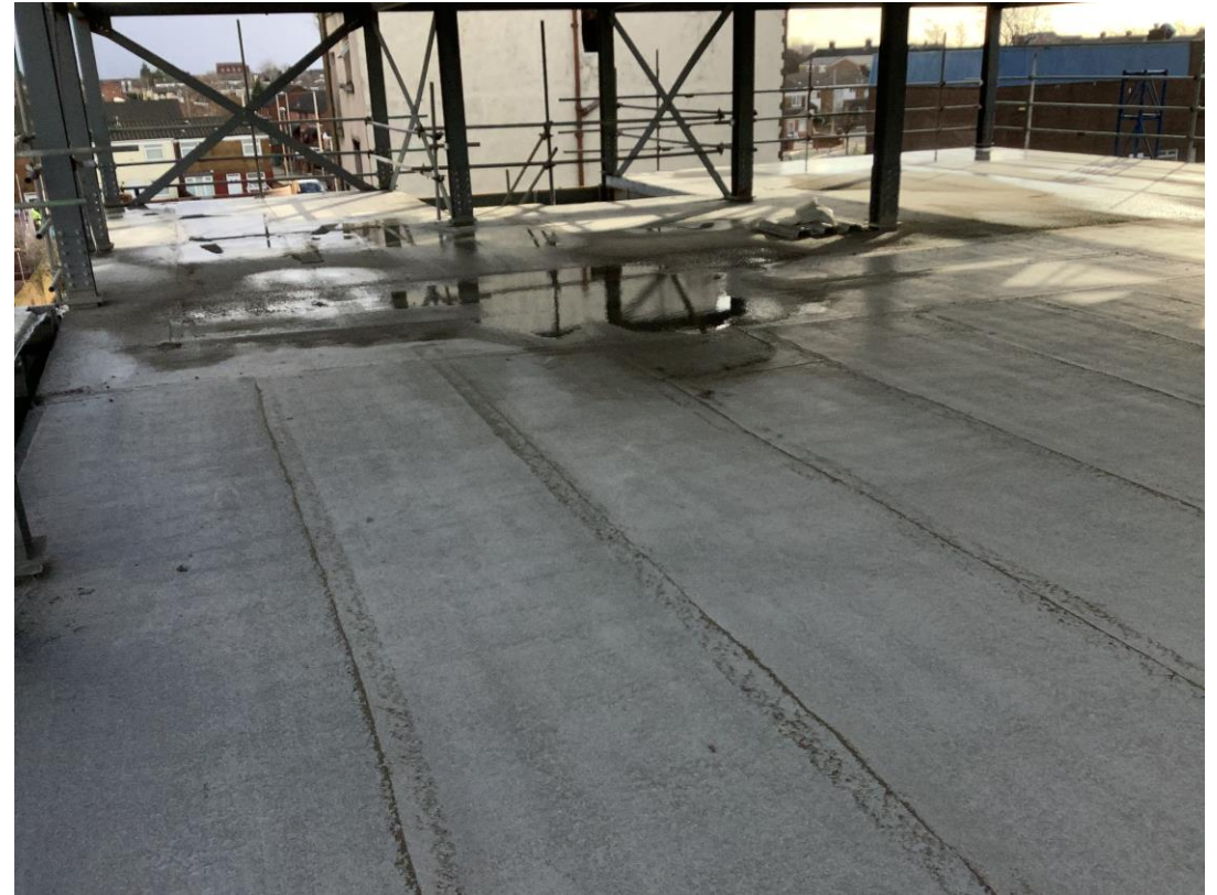
Commercial block - Concrete floor slab
