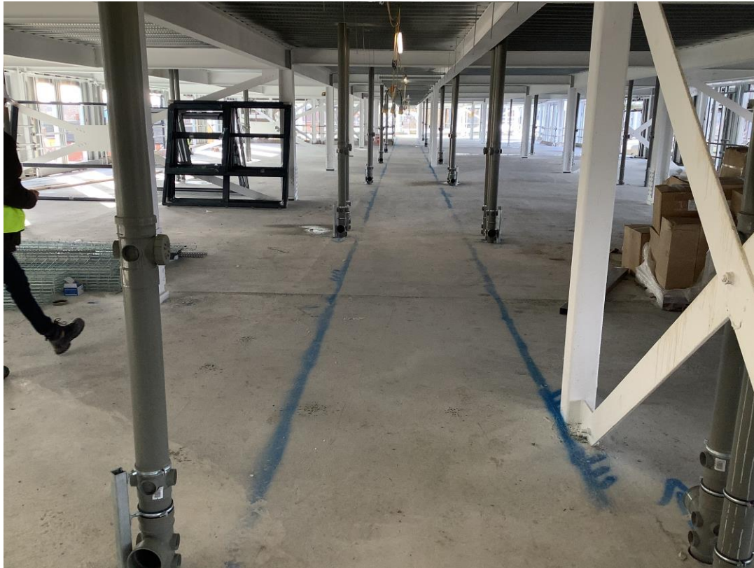
Residential wing - Setting out partitions
