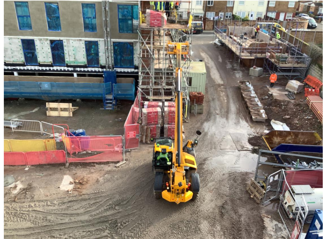
Inner courtyard - General site activity
