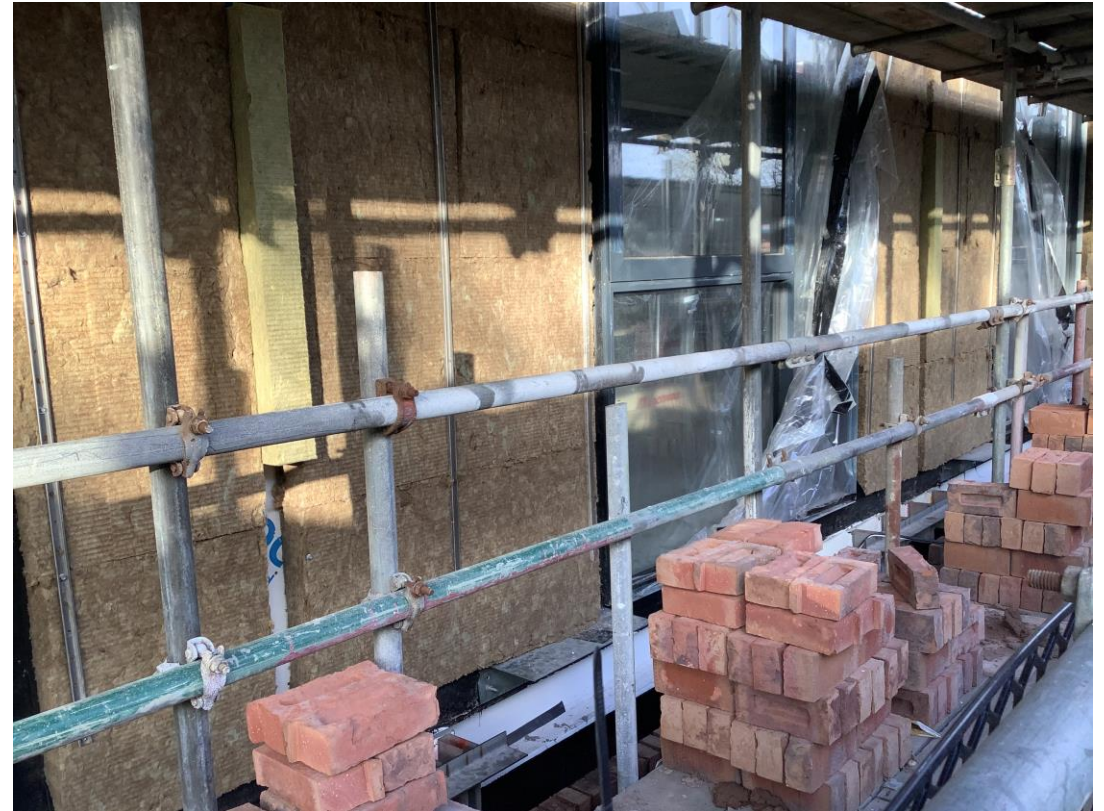
Student wing - External wall insulation ongoing
