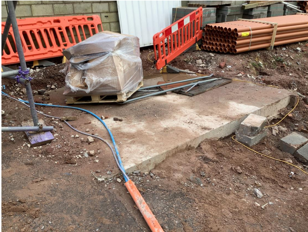
External concrete base
