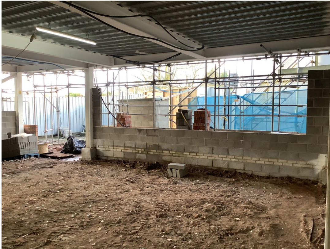
Student wing - Low level blockwork progress
