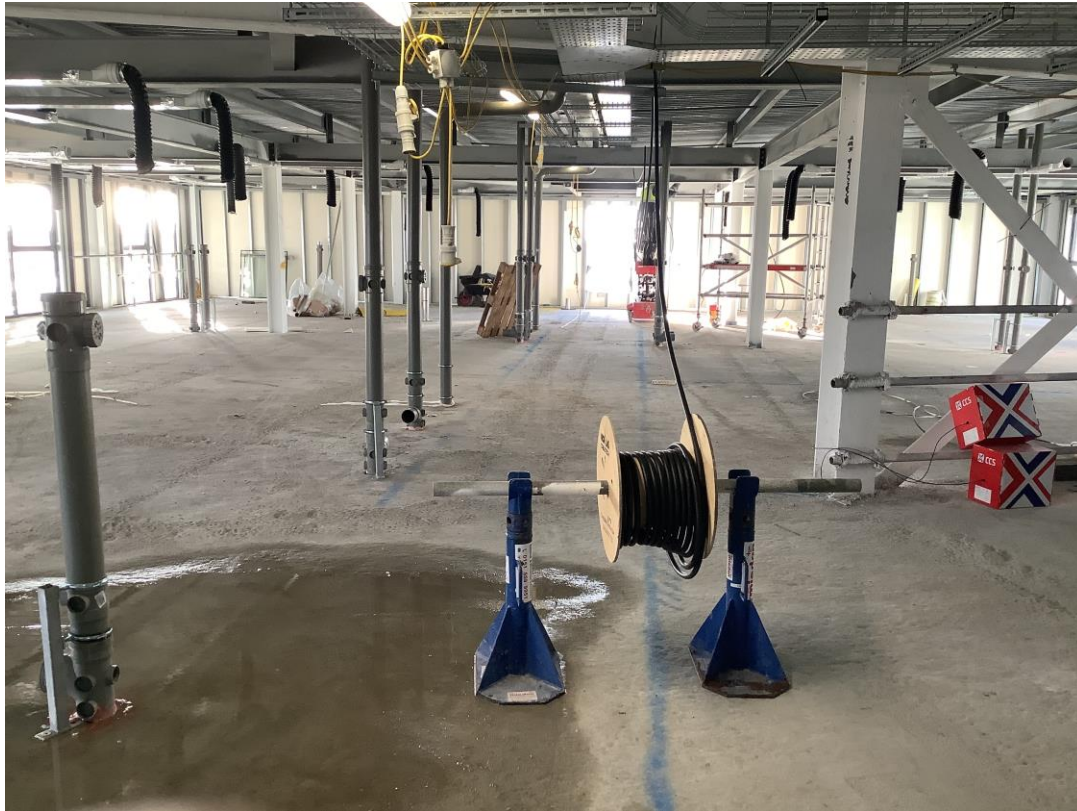
Student wing - First fix Electrical works
