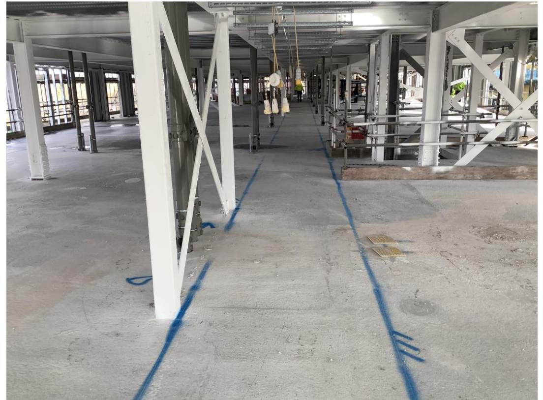
Residential wing - Setting out partitions
