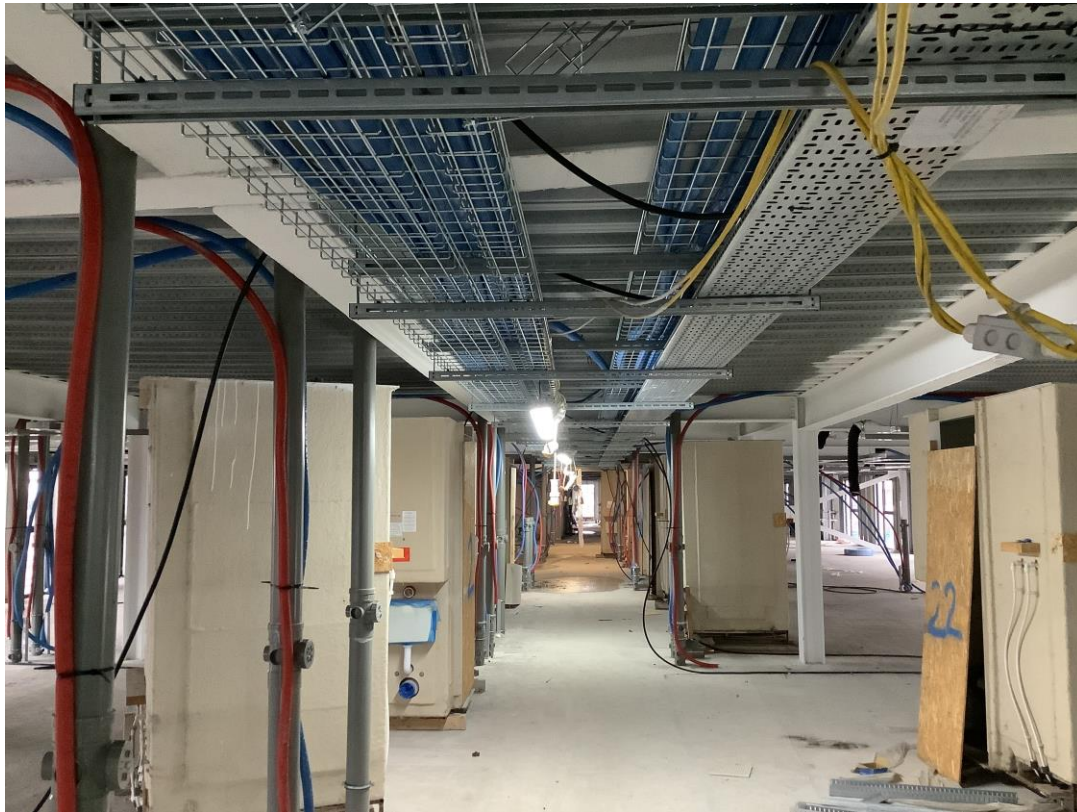
Student wing - First fix Mechanical & Electrical works
