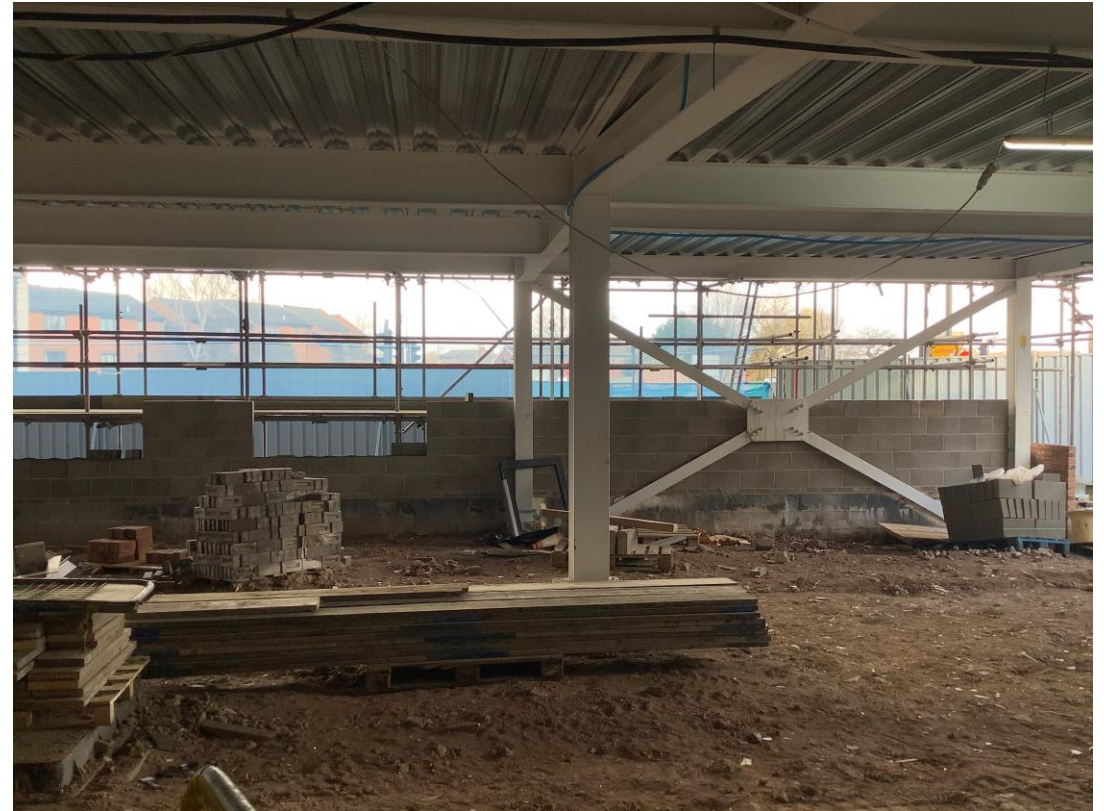
Student wing - Low level blockwork progress
