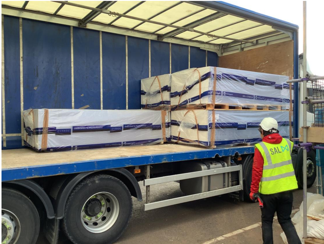
Materials delivery - Plasterboard
