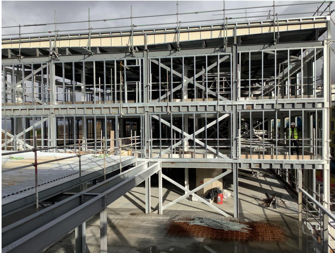
Residential wing - Steel frame structure and SFS & weatherboard
