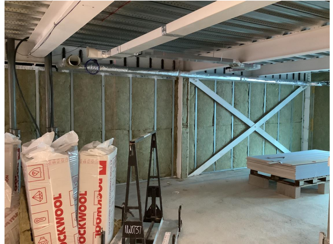
Student wing - Gable end insulation
