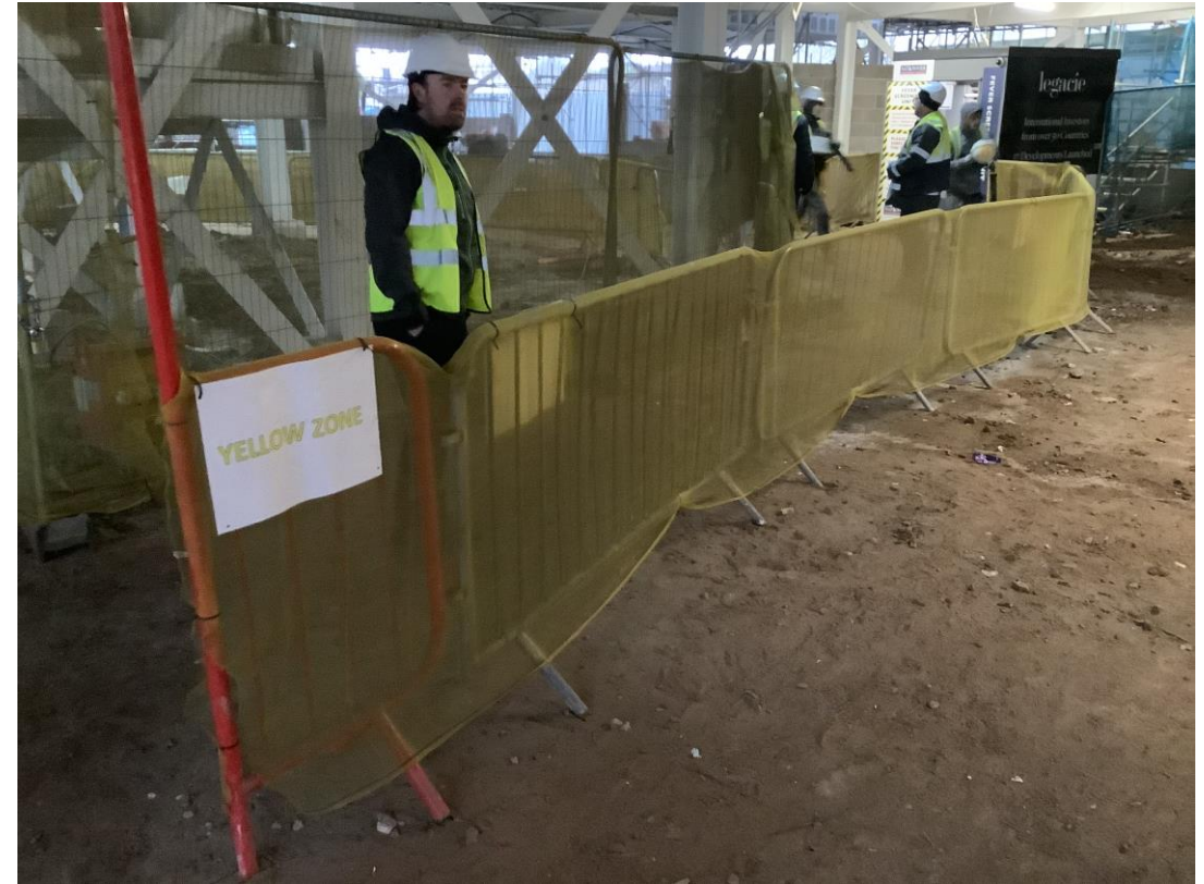
Site barriers being utilised
