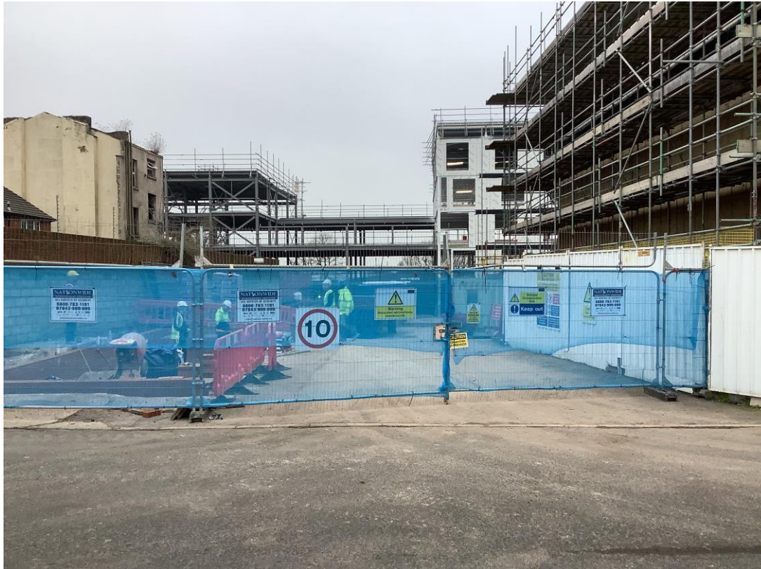
Walker Street - Secure site access for plant and deliveries
