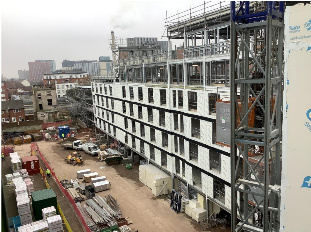
Inner courtyard - General site activity
