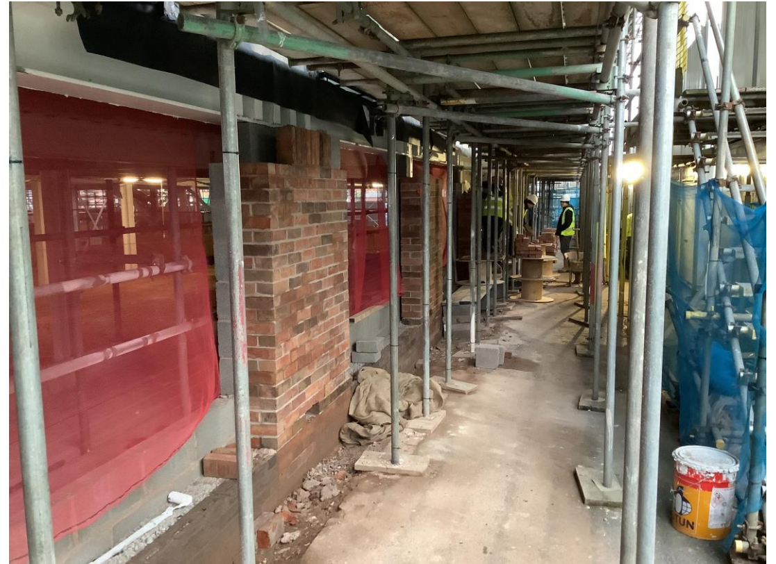
Student wing - Cavity wall brickwork
