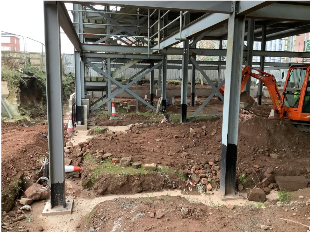
Commercial block - Under ground drainage and ground floor beams
