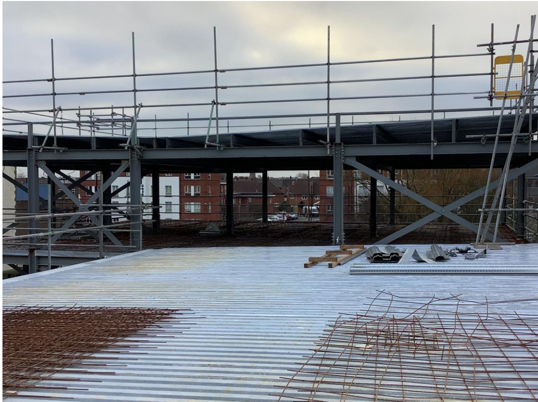
Commercial block - Upper suspended steel floor structure
