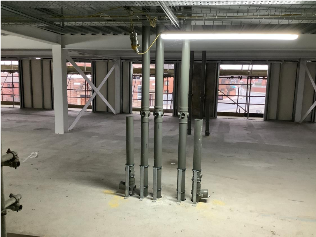
Residential wing - First fix Mechanical works
