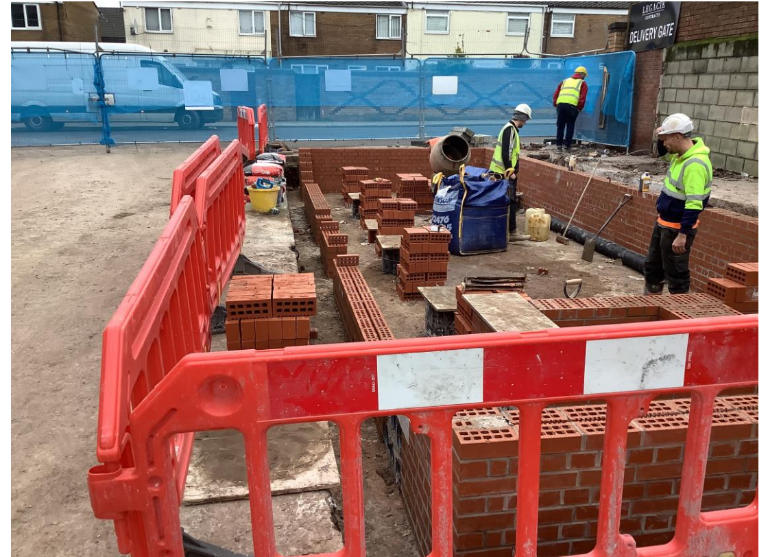
Brickwork progress to sub-station
