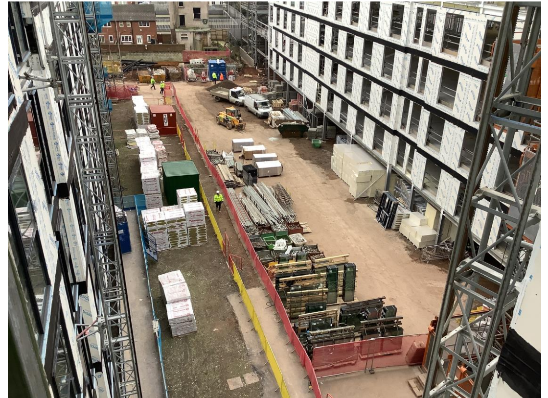
Inner courtyard - General site activity
