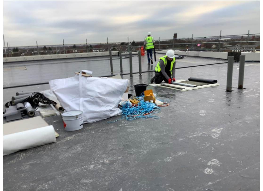
Student Wing - Flat roof membrane installed
