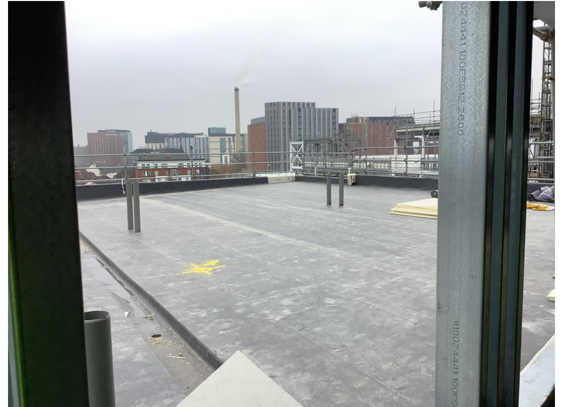
Student Wing - Flat roof membrane installed
