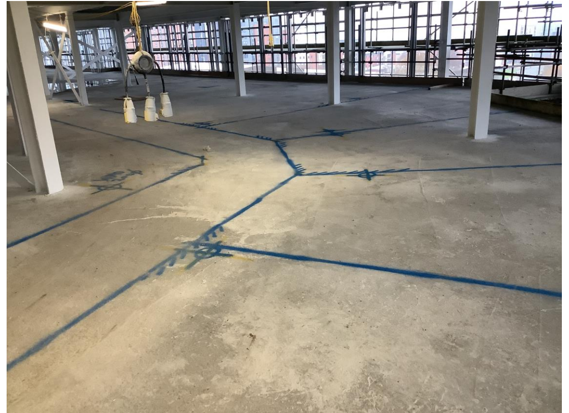
Residential Wing - Setting out partitions
