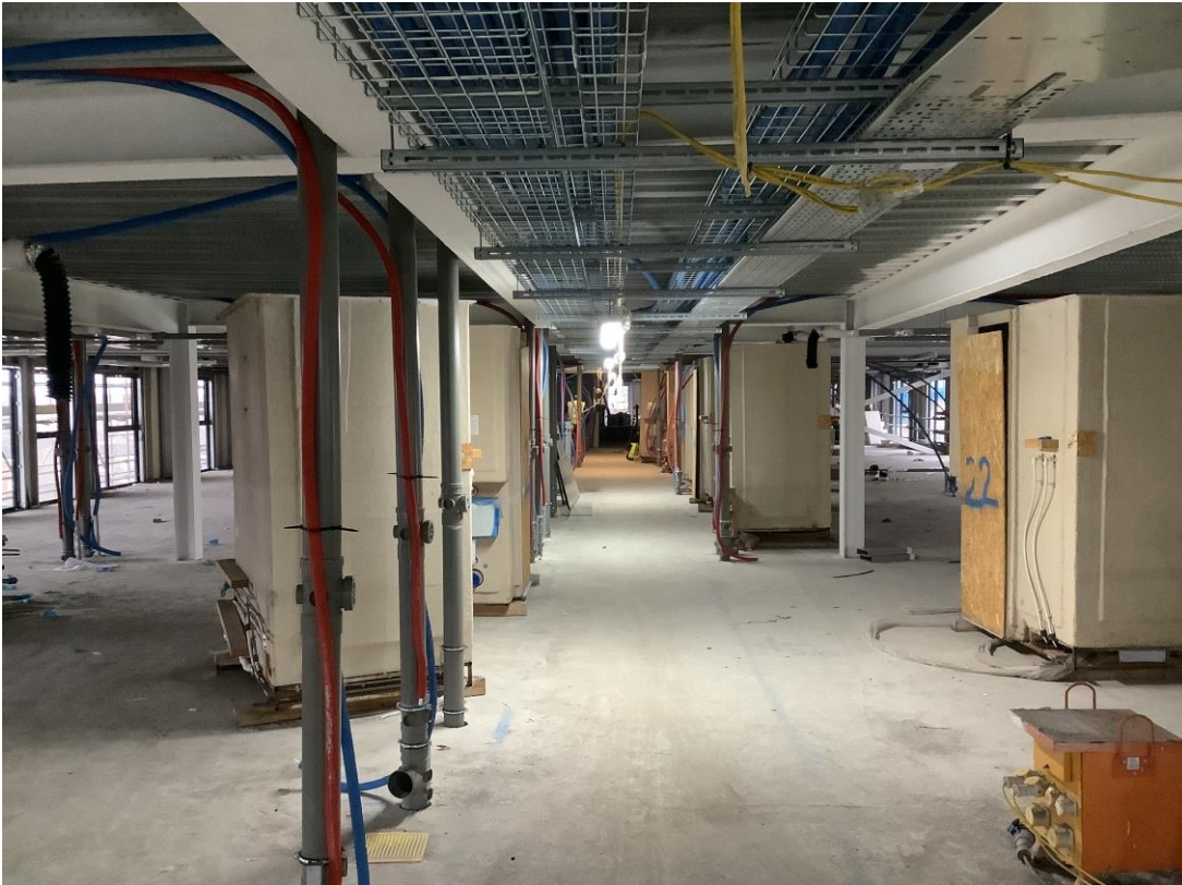
Student wing - First fix Mechanical & Electrical works
