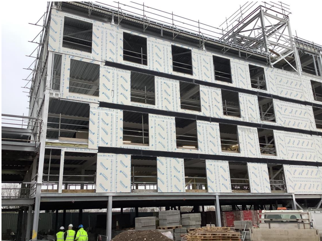
Inner courtyard view - Steel frame structure and SFS & weatherboard
