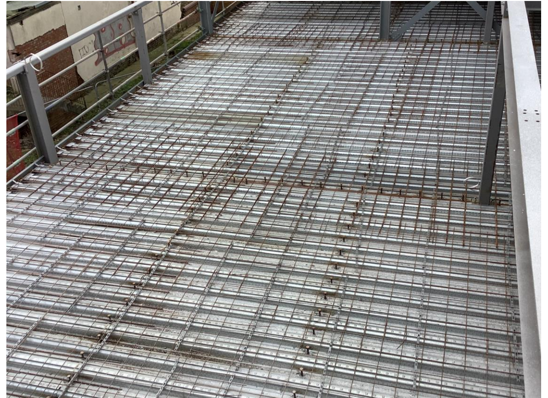
Commercial block - Upper suspended steel floor structure
