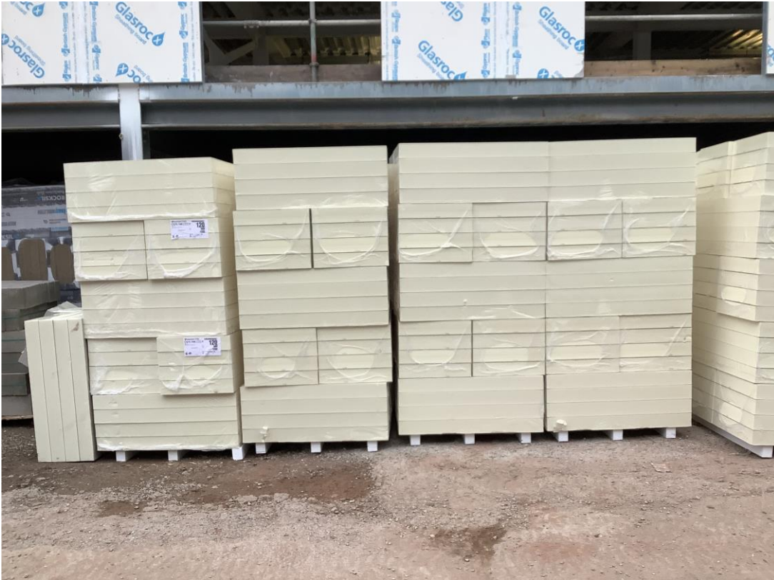
Material storage - Insulation
