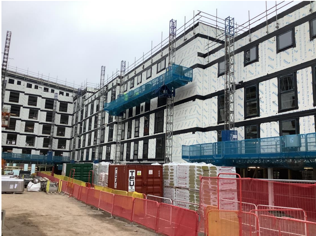
Inner courtyard view - SFS & weatherboard, windows and mast climbers
