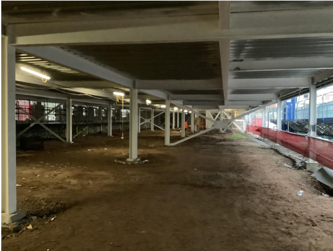
Undercroft parking area fire coating
