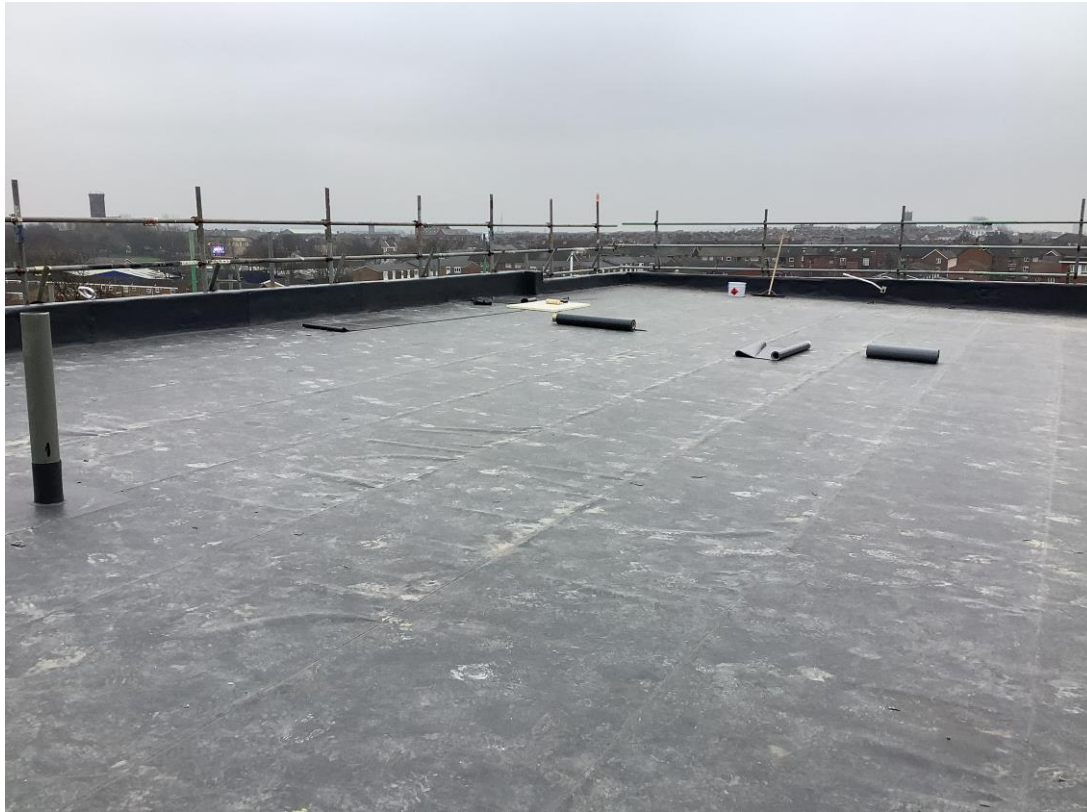
Student Wing - Flat roof membrane installed
