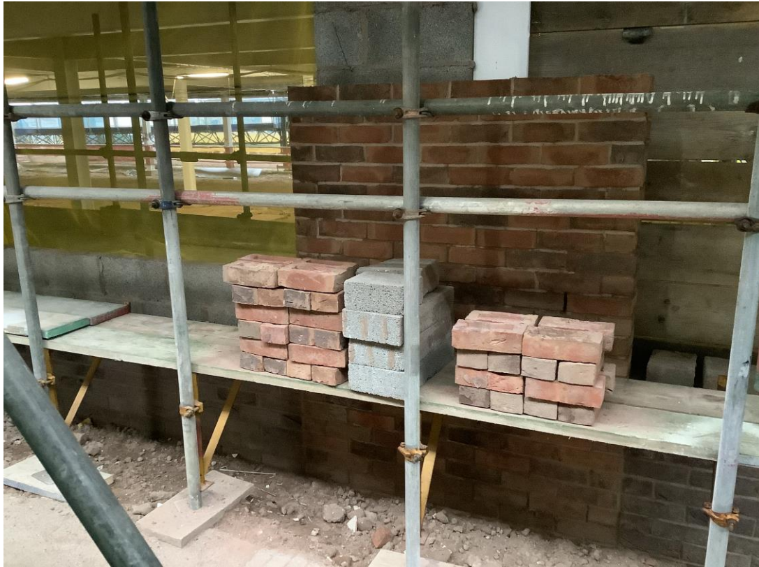
Student wing - Cavity wall brickwork
