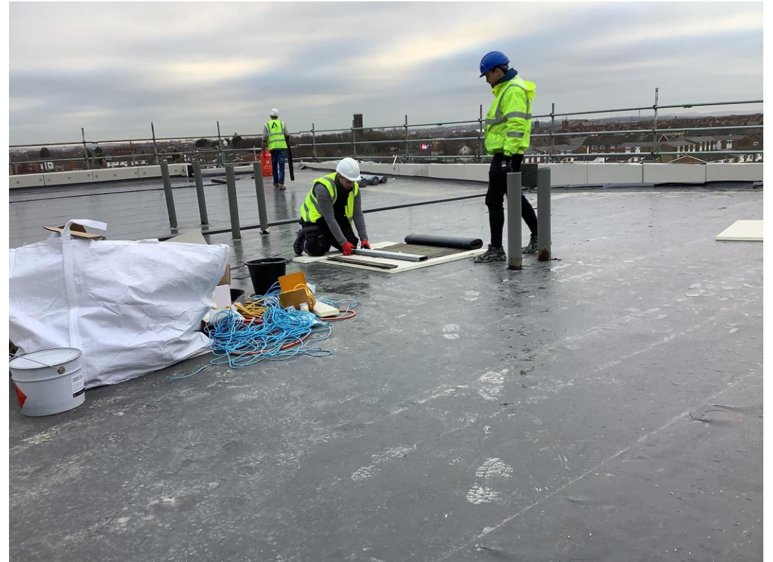
Student Wing - Flat roof membrane installed
