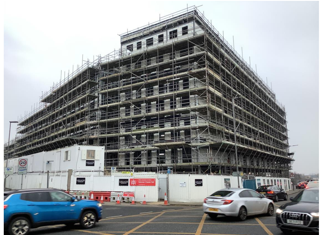
West Derby Road - Site view
