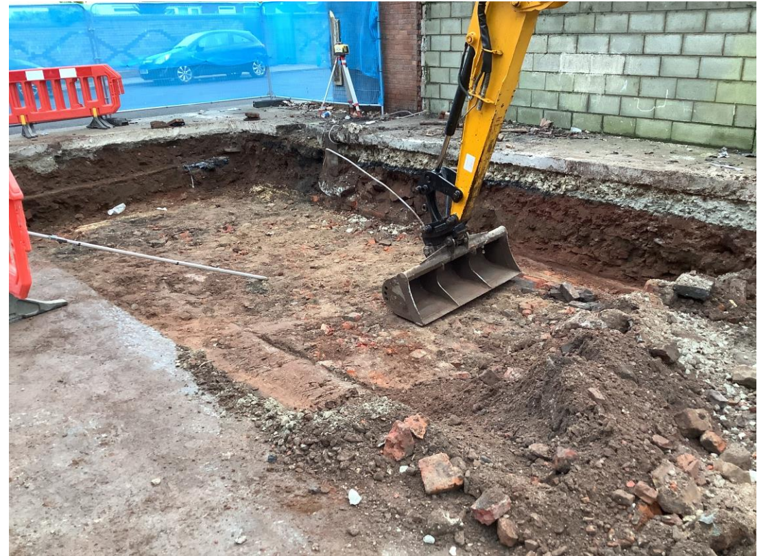
Excavation works to form sub-station
