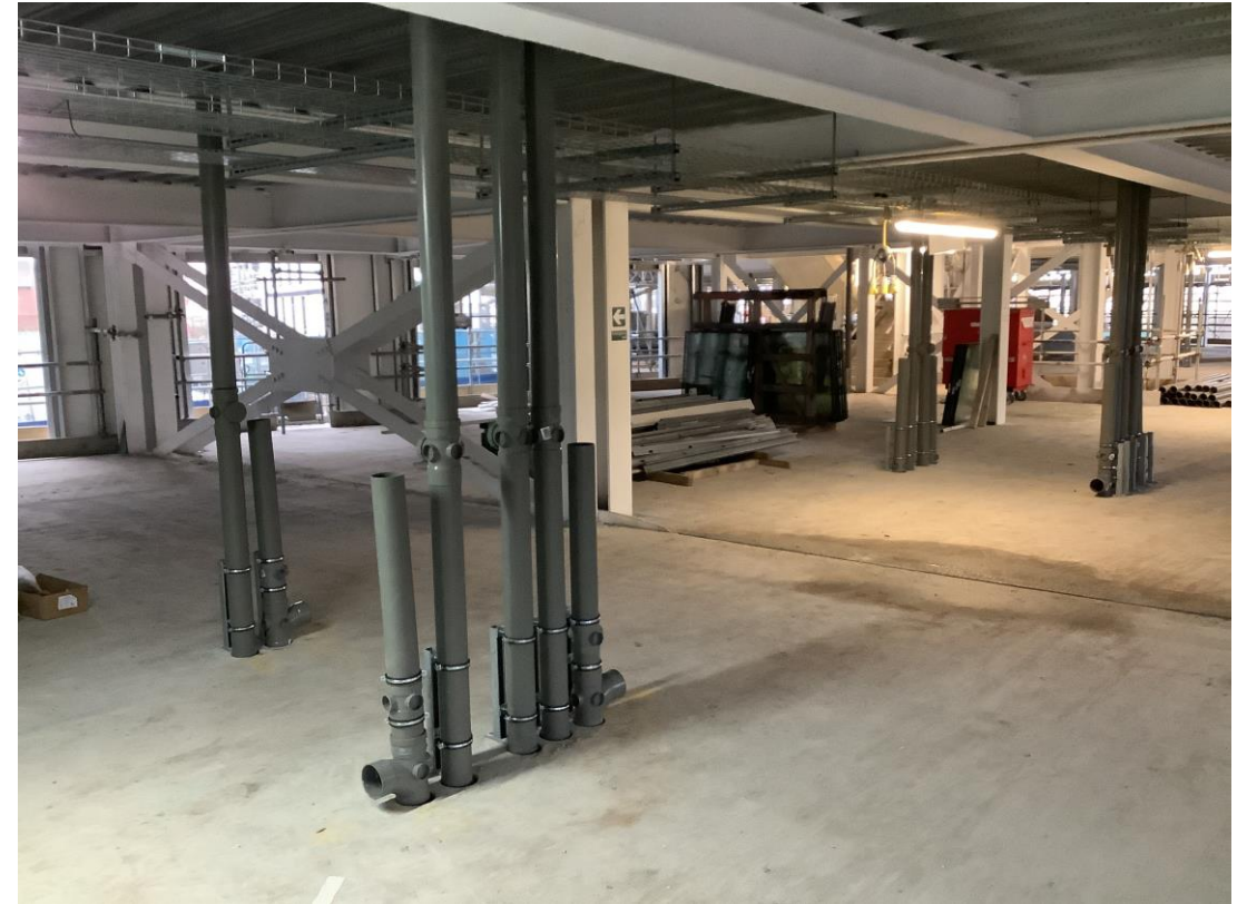
Residential wing - First fix Mechanical works
