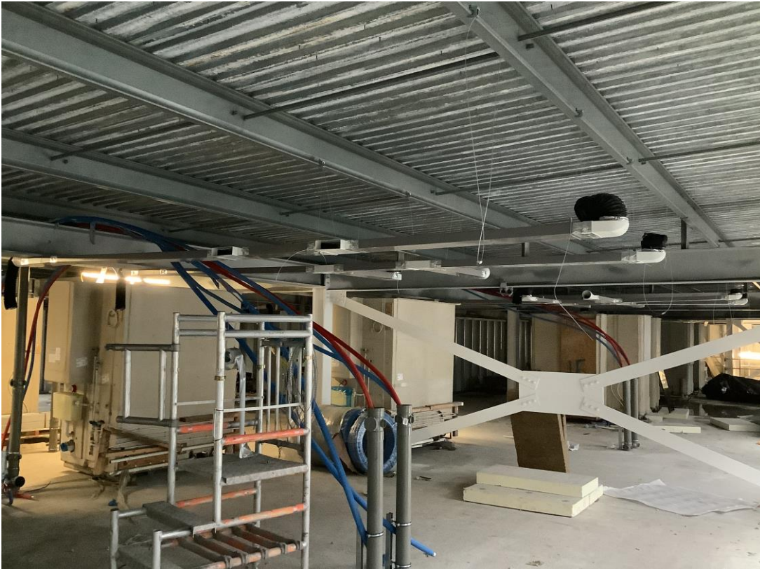
Student wing - First fix Mechanical ducting
