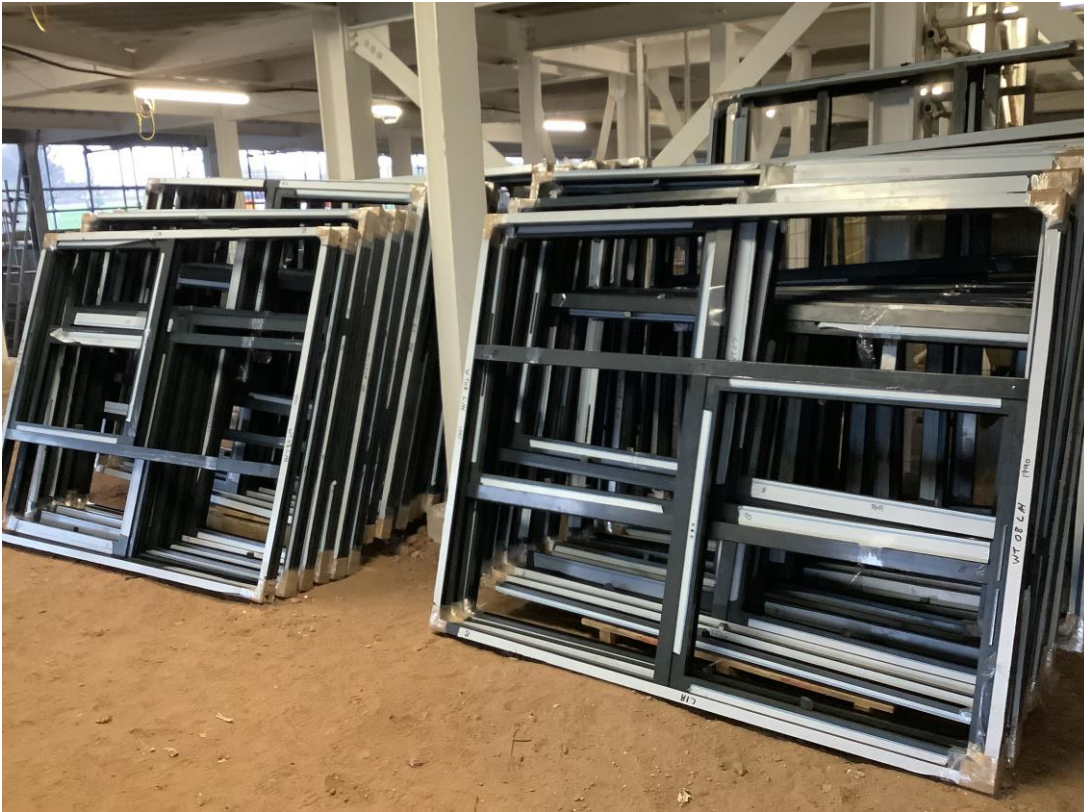
Material storage - Window frame
