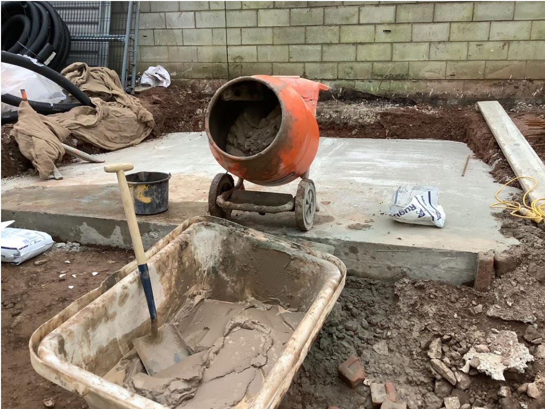
Concrete base construction
