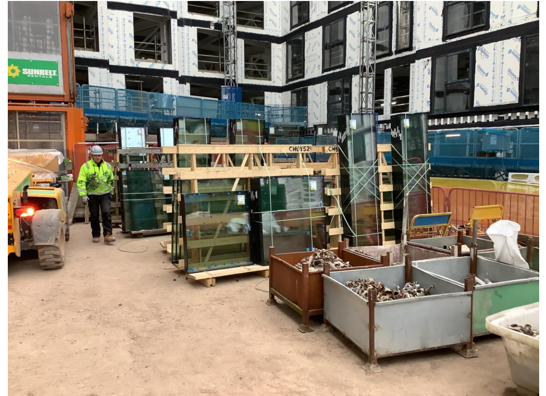
Material storage - Glazing units
