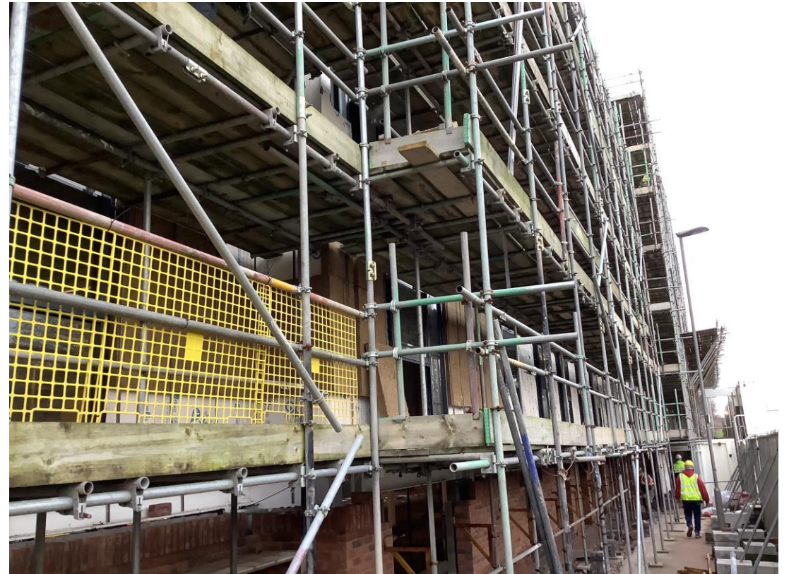
Student wing - External wall insulation
