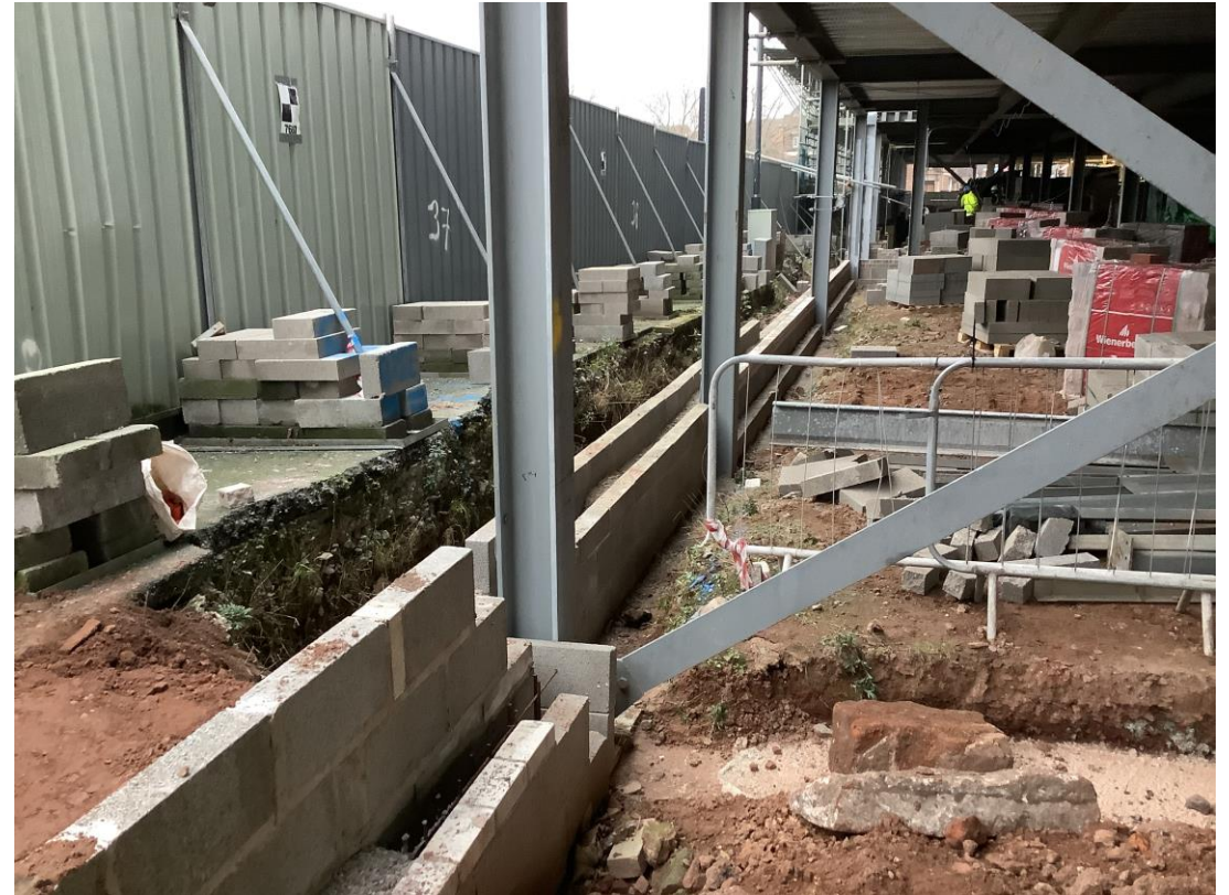
Commercial block - Retaining wall blockwork
