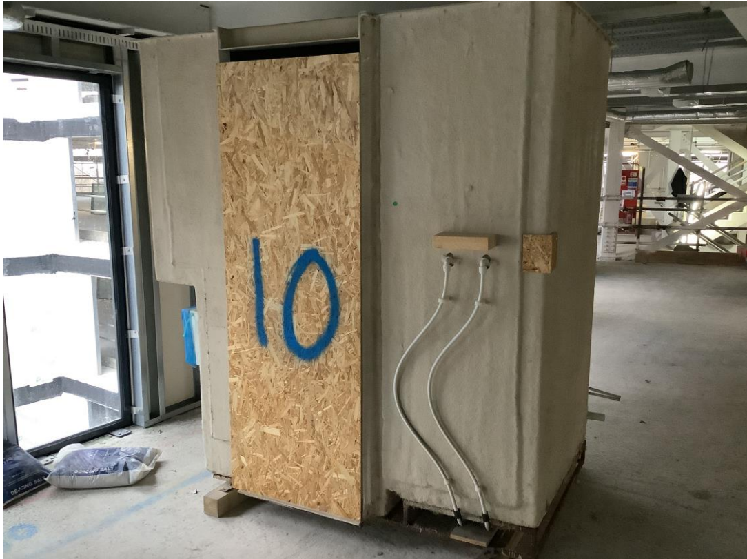
Residential wing - Pod testing complete
