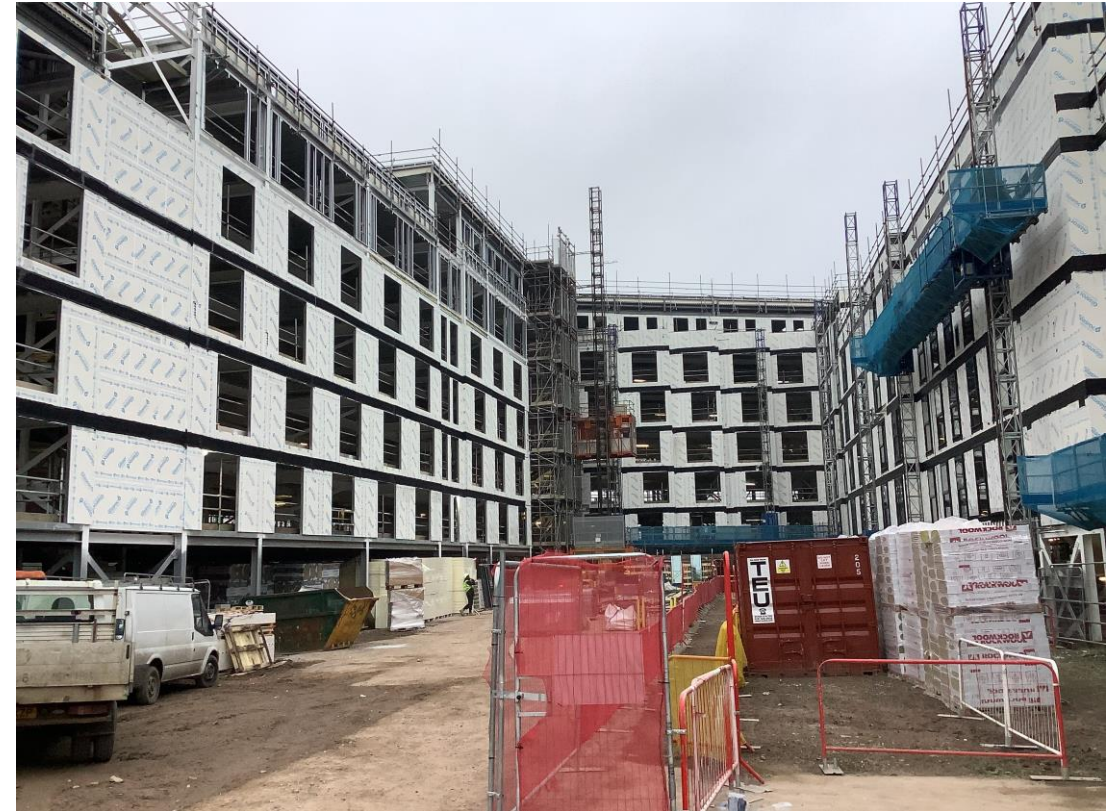
Inner courtyard - General site view
