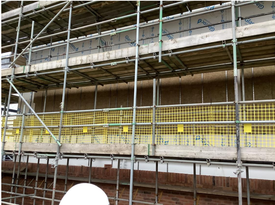
Student wing - External wall insulation
