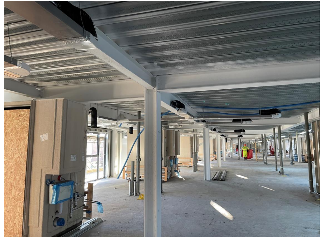
Mechanical installations commenced to student wing
