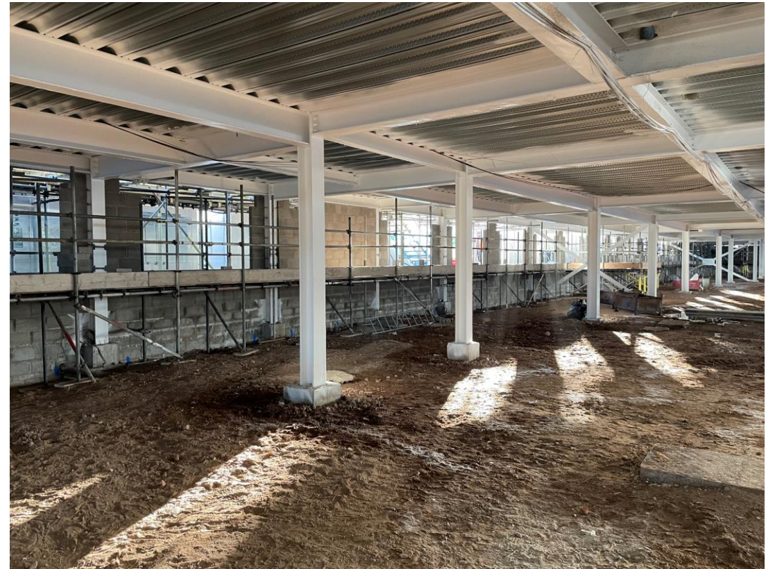
Construction of external wall blockwork to undercroft parking area
