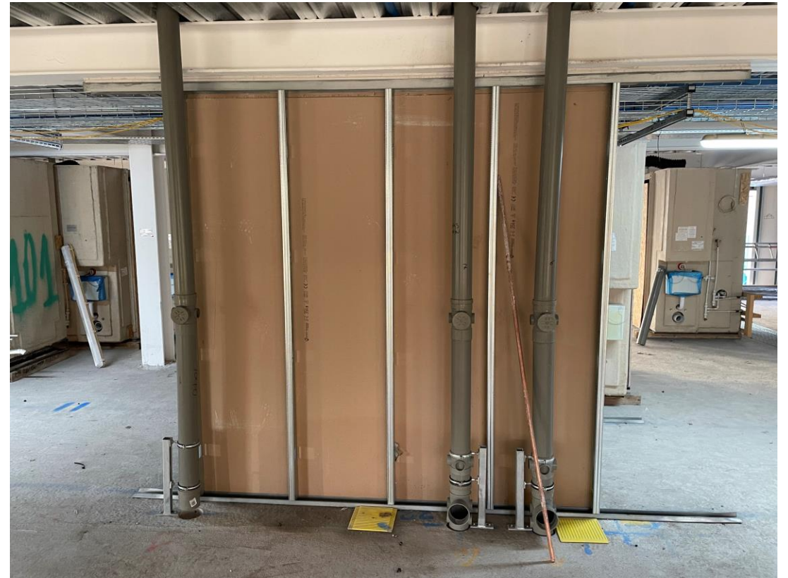
Metal stud and plaster boarded partition wall mock-up – Student wing
