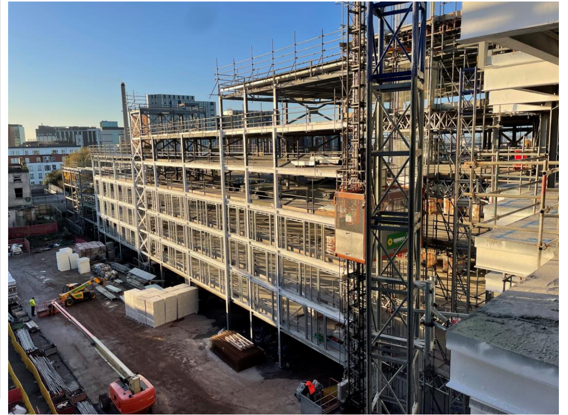
Steel frame structure – Residential wing
