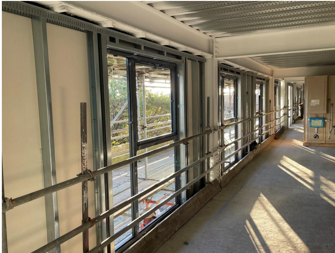
Installation of window units commenced – Student wing
