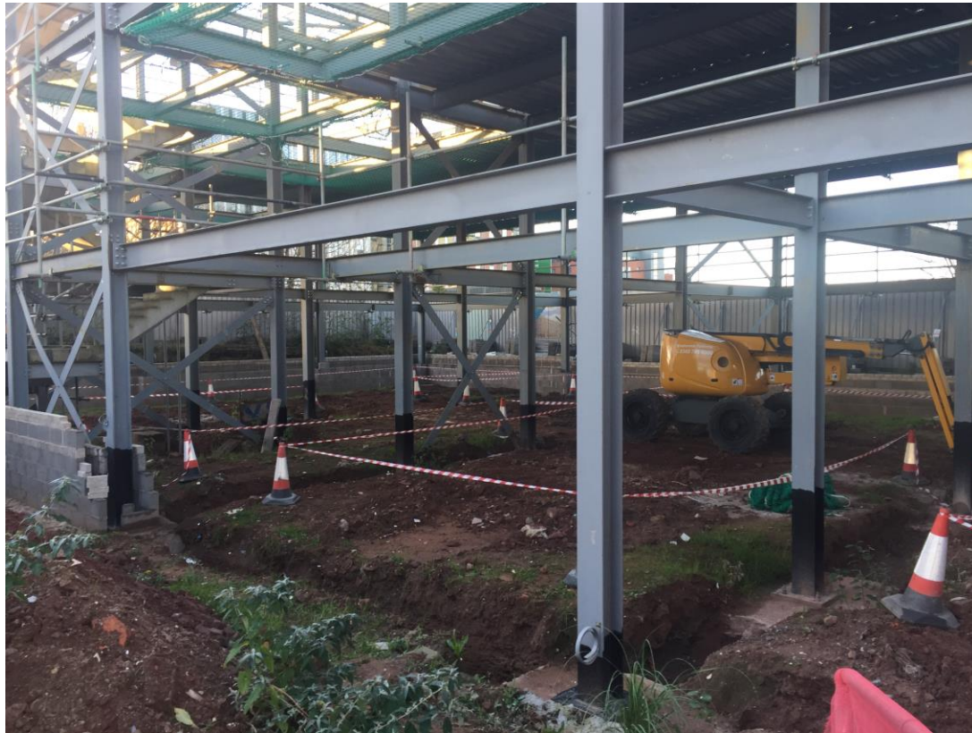
Installation of under ground drainage and ground floor beams on-going
