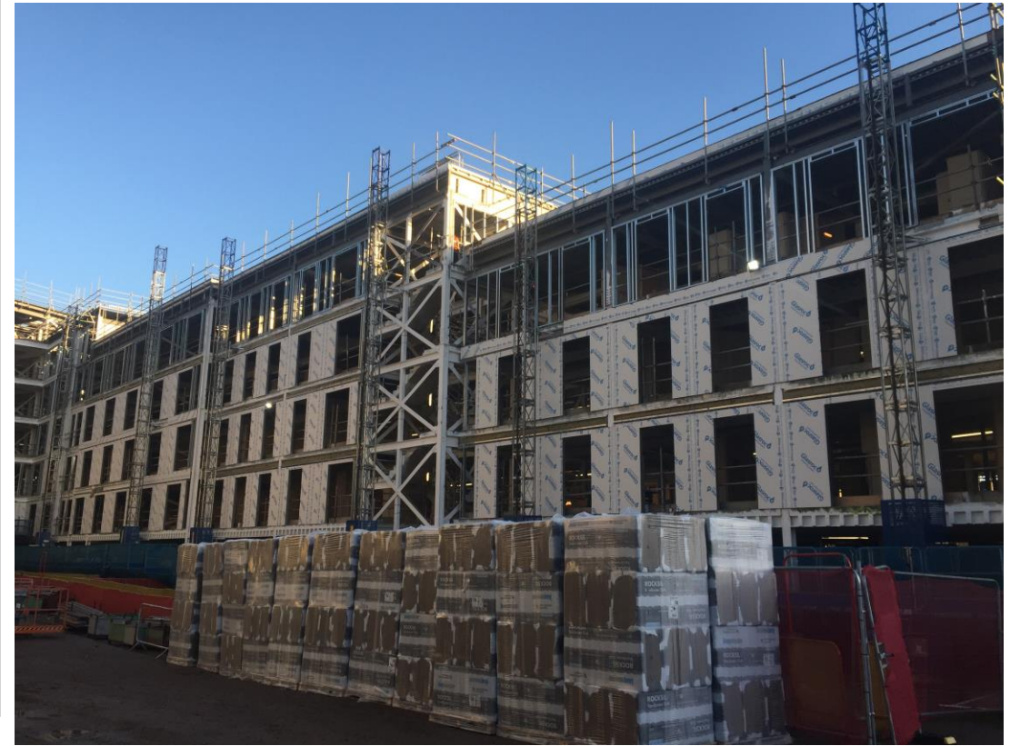
Inner courtyard view, Steel framework structure, SFS & weatherboard and mast climbers
