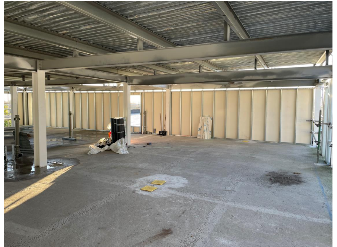
SFS & weatherboarding to upper floors – Student wing
