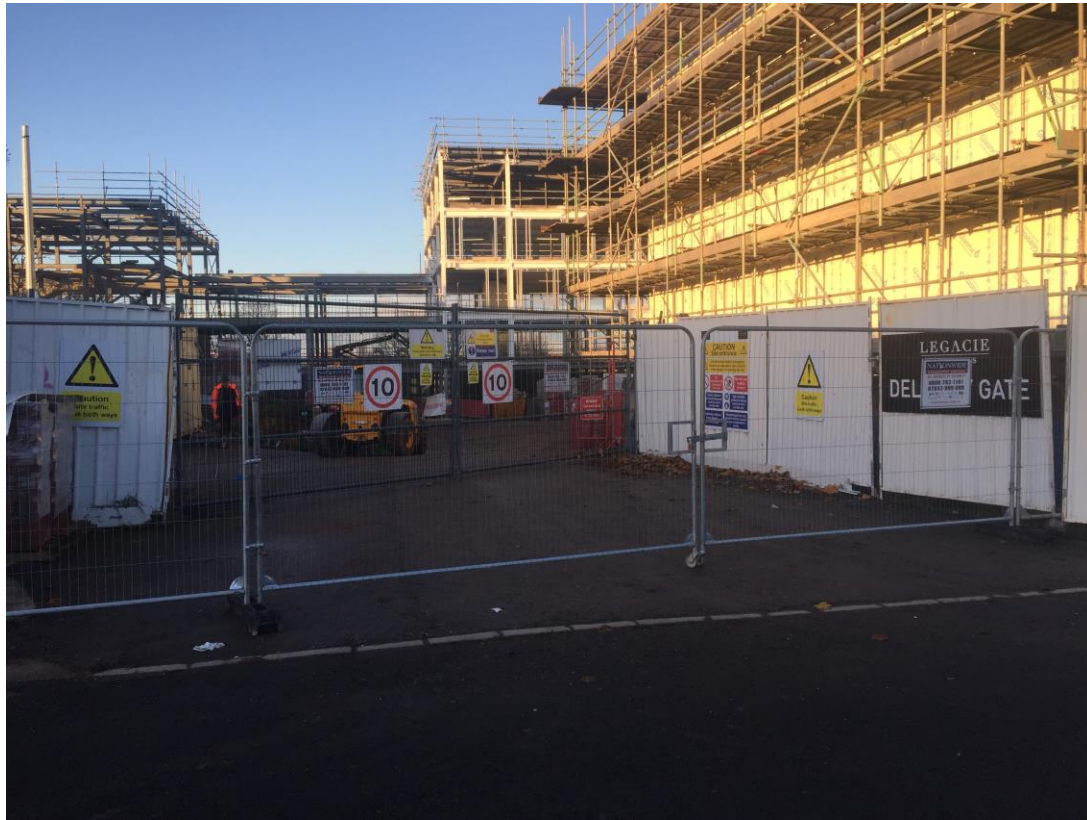
Secure site access for plant and deliveries
