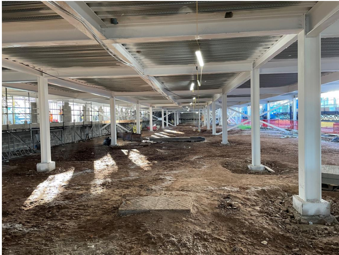
Undercroft parking area
