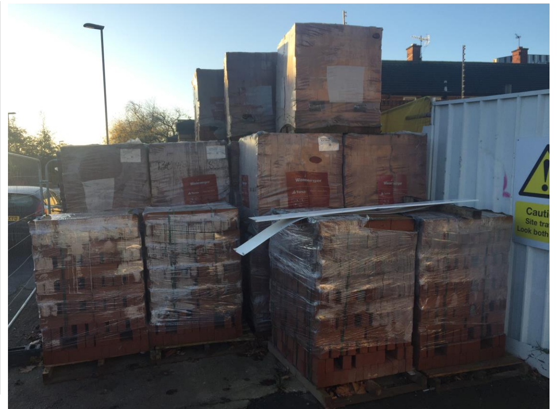
Material storage – Red Brick
