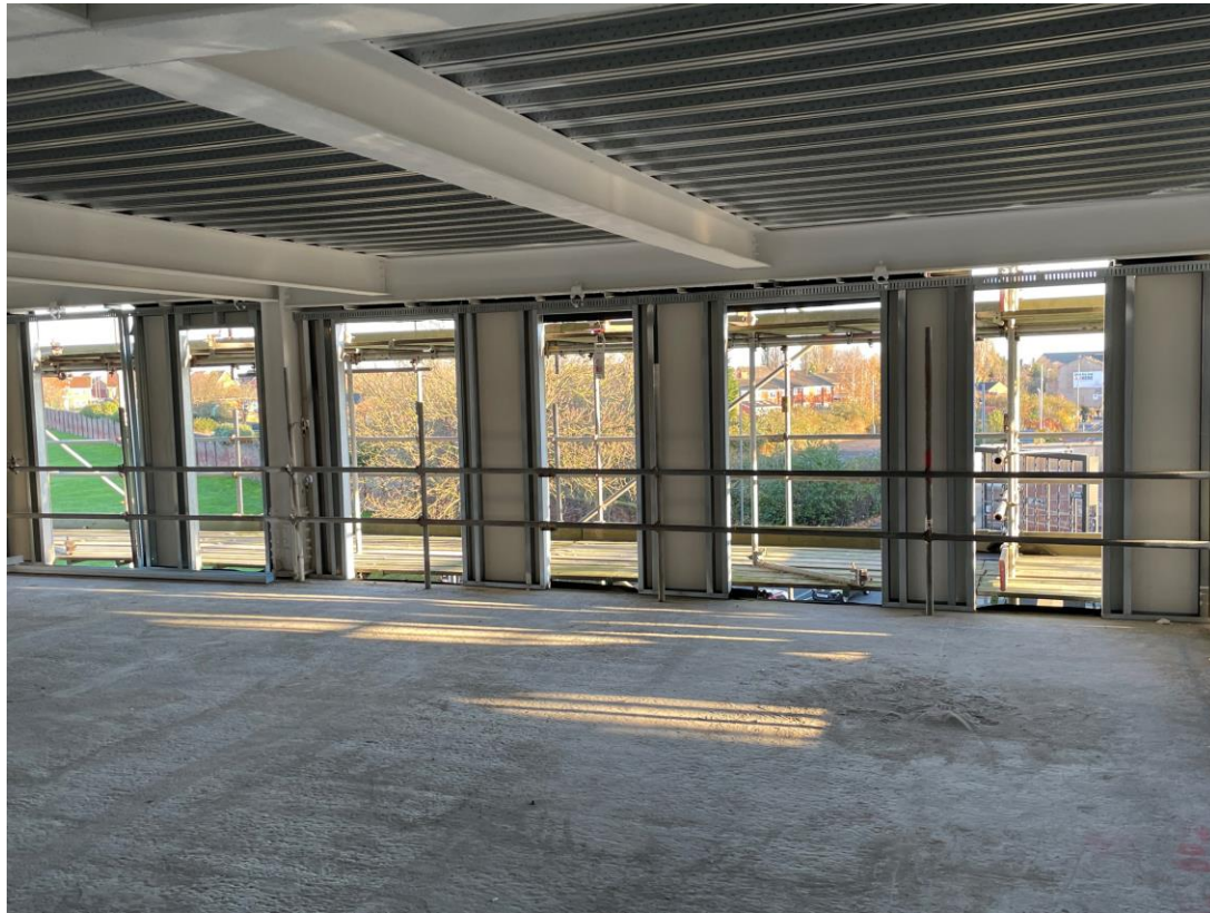
SFS & weatherboarding on-going – Student wing
