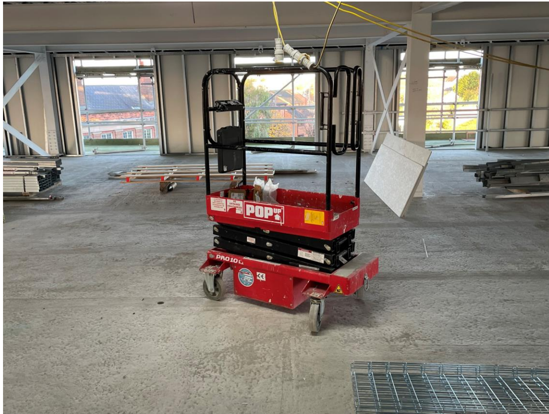
Mobile elevating work platform (MEWP) observed – Student wing
