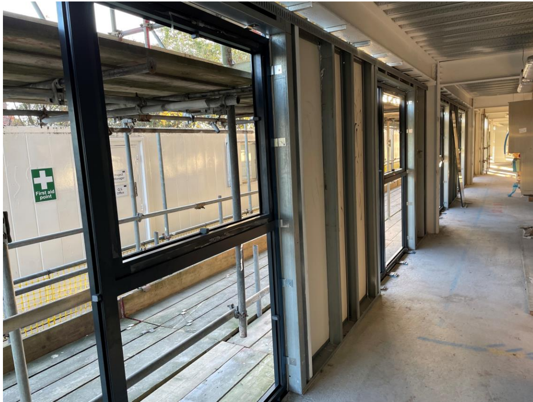
Installation of window units commenced – Student wing
