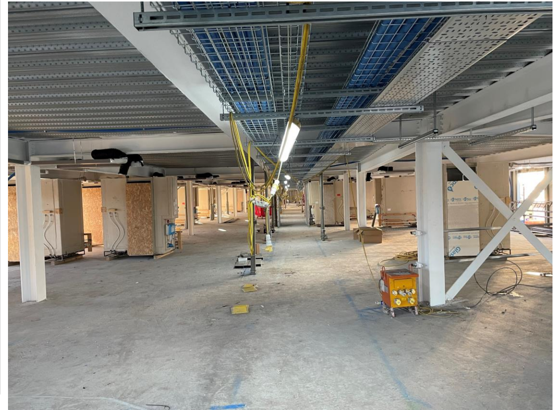
Installation of pipe runs to new containment commenced – Student wing
