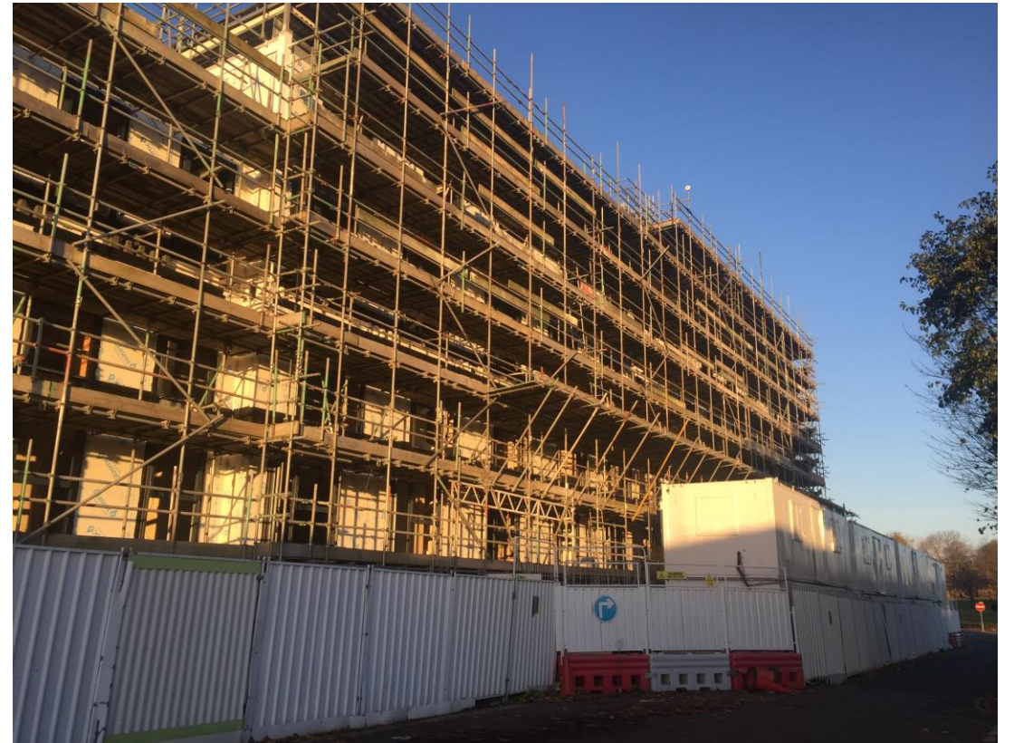
Walker Street - Site view
