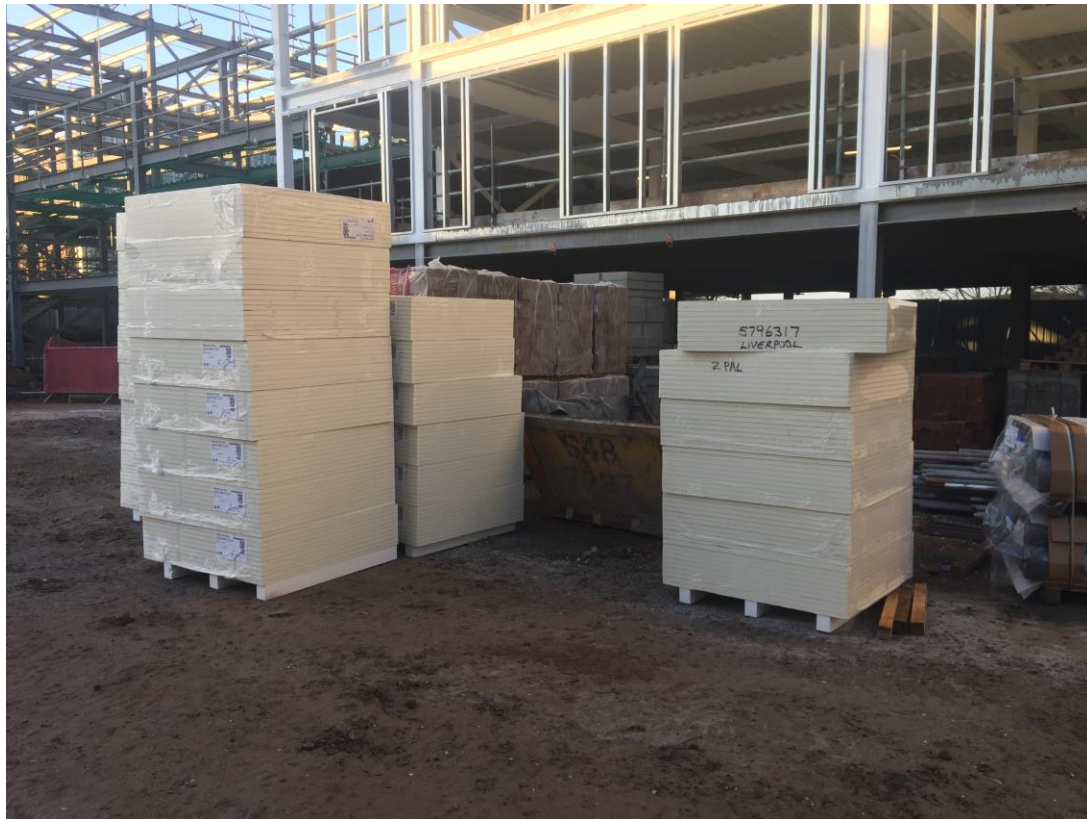
Material storage - Insulation
