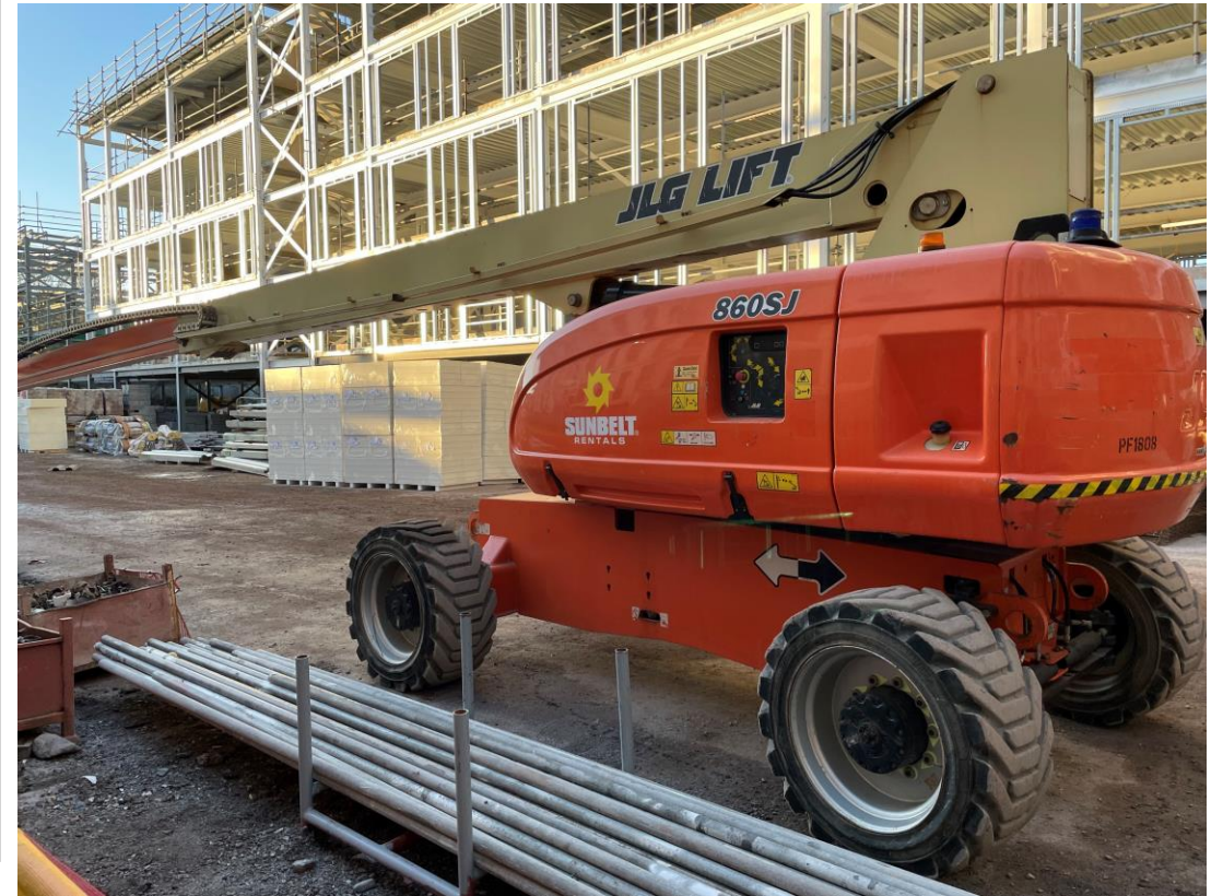
Site access plant
