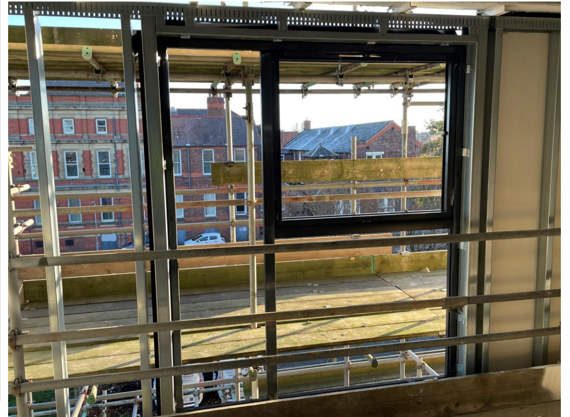
Installation of window units commenced – Student wing
