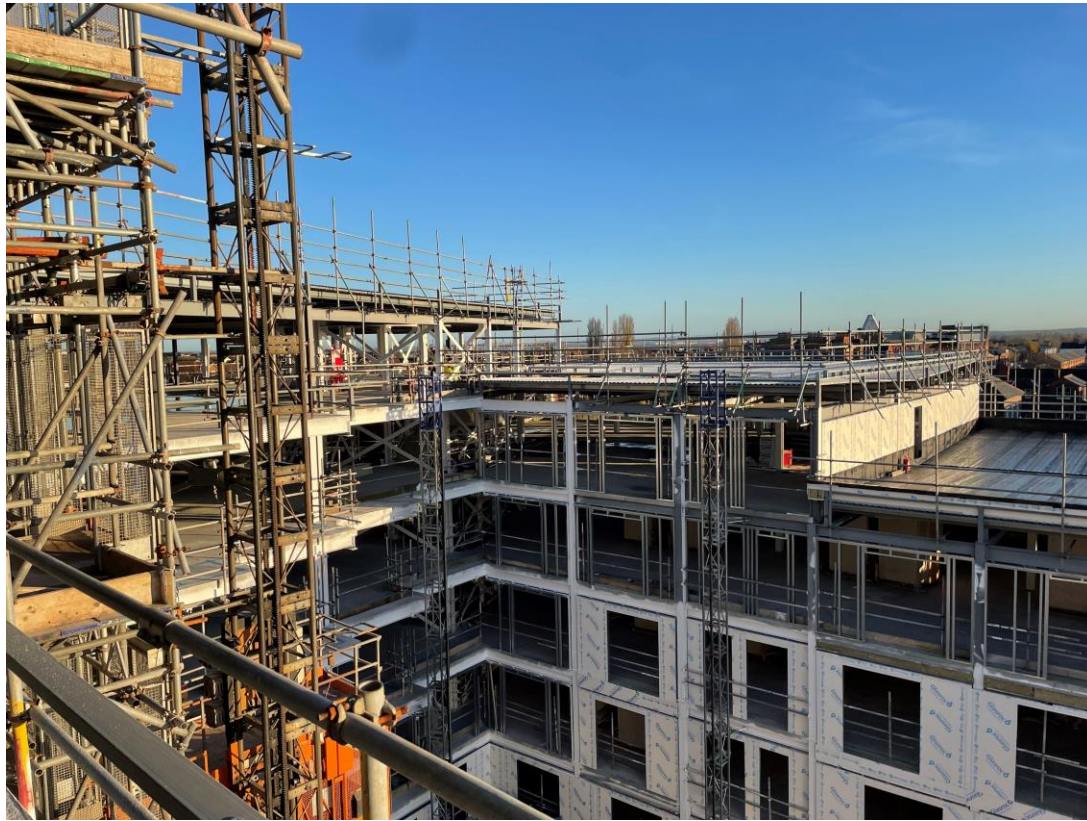
Metal decking structure and waterproofing to roof – Student wing
