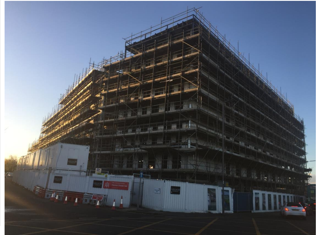
West Derby Road - Site view
