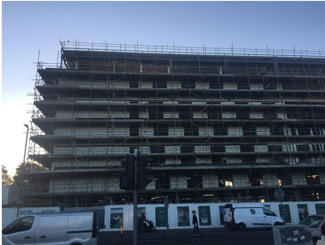
West Derby Road - Site view
