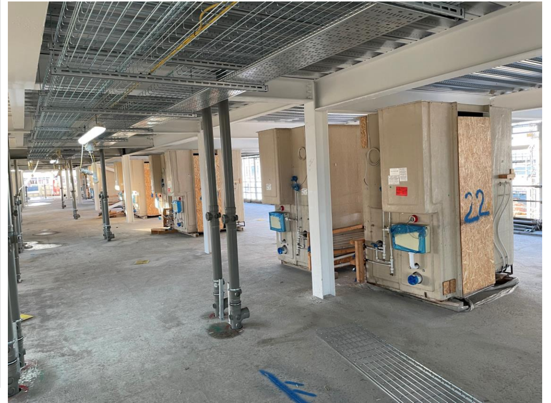
Above ground drainage installation to upper floors – Student wing
