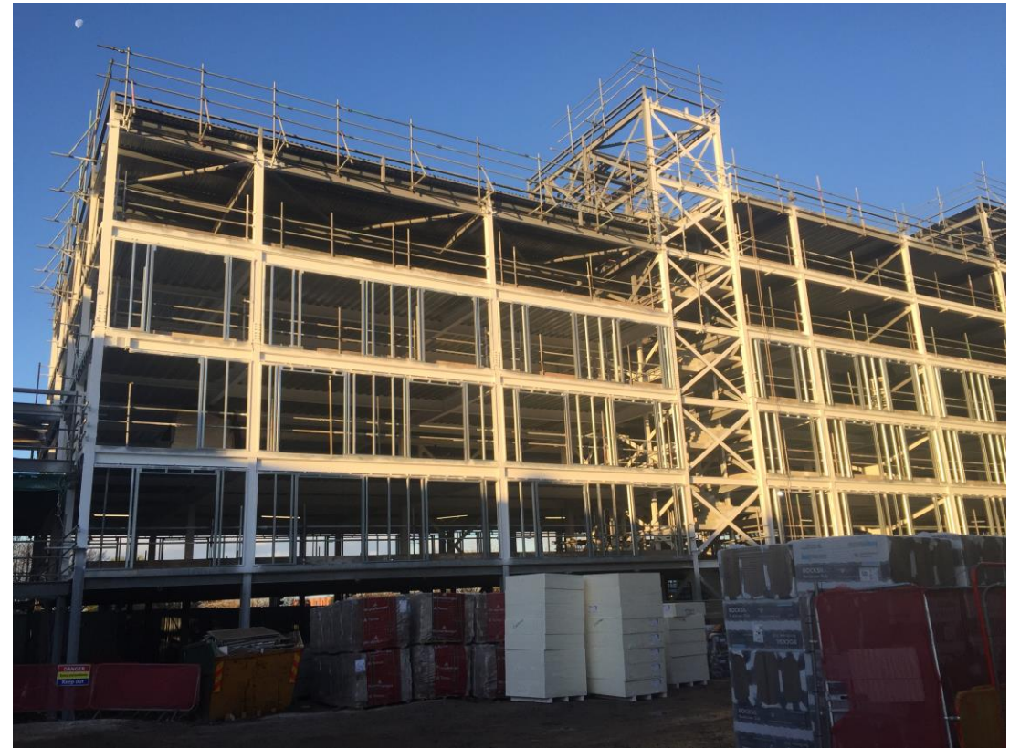
Steel frame structure – Residential wing
