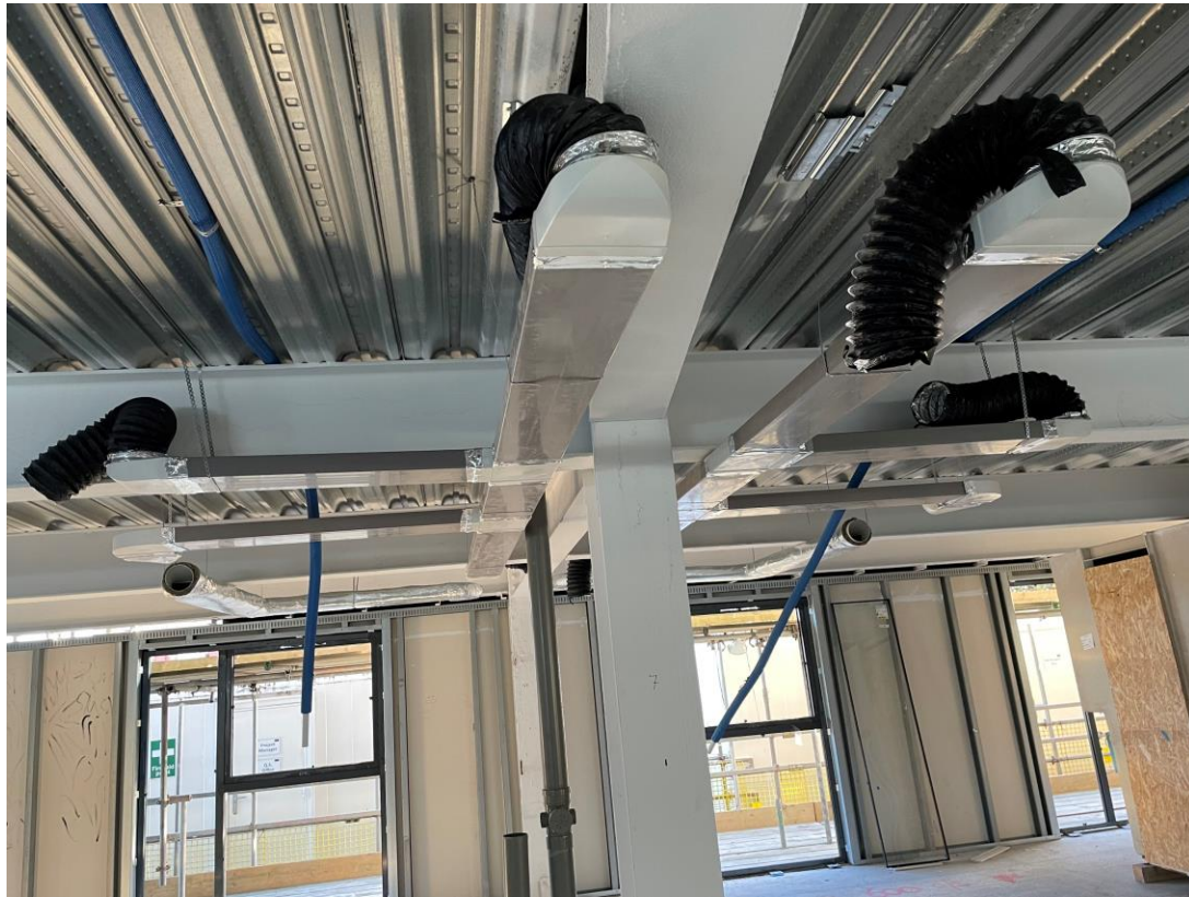
Mechanical installations commenced to student wing
