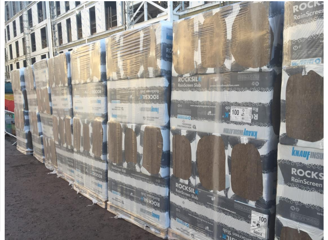
Material storage – Rainscreen slab
