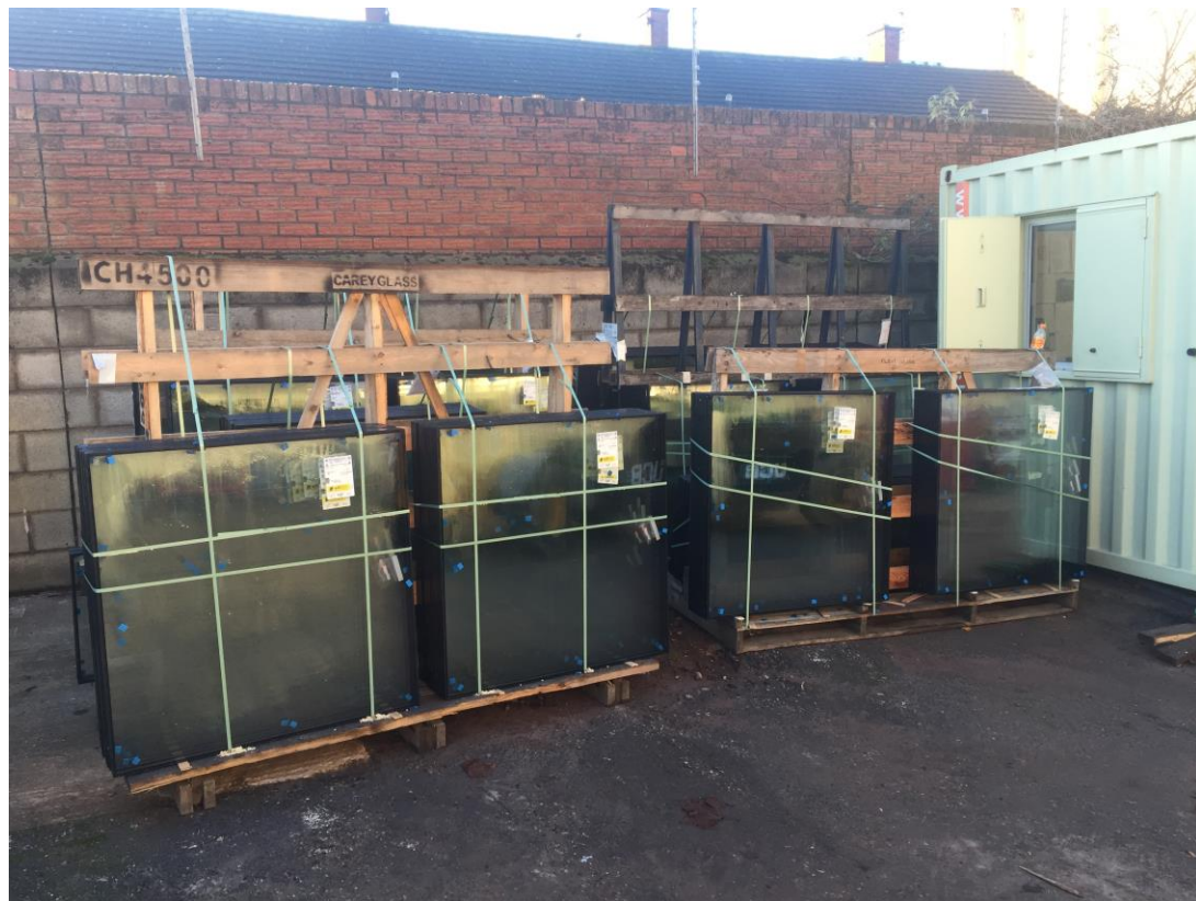
Material storage – Glazing Panels
