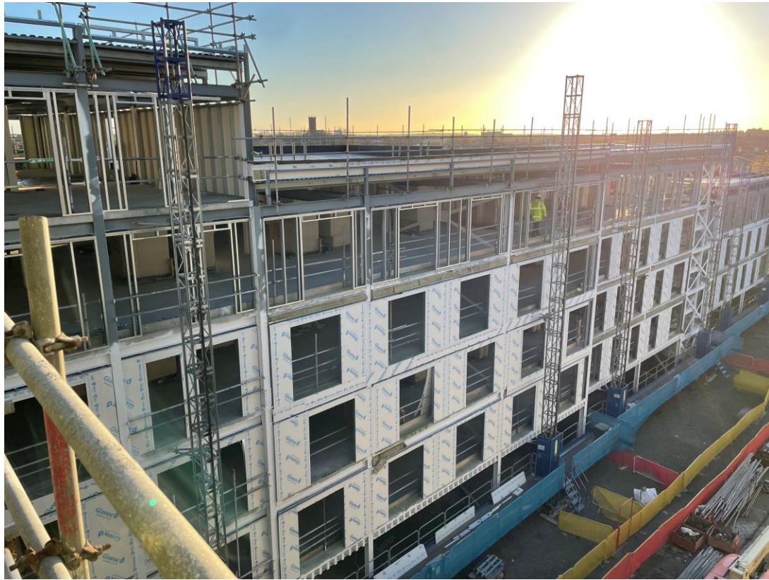
Steel framework structure, SFS & weatherboard and mast climbers
