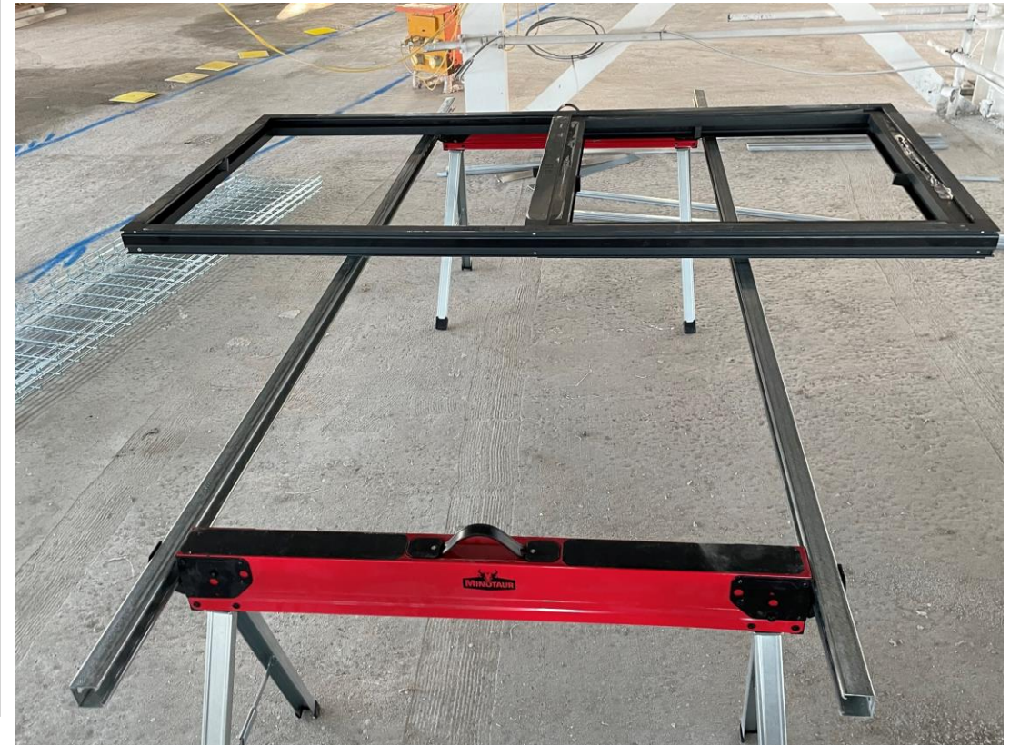
Installation of window units commenced – Student wing
