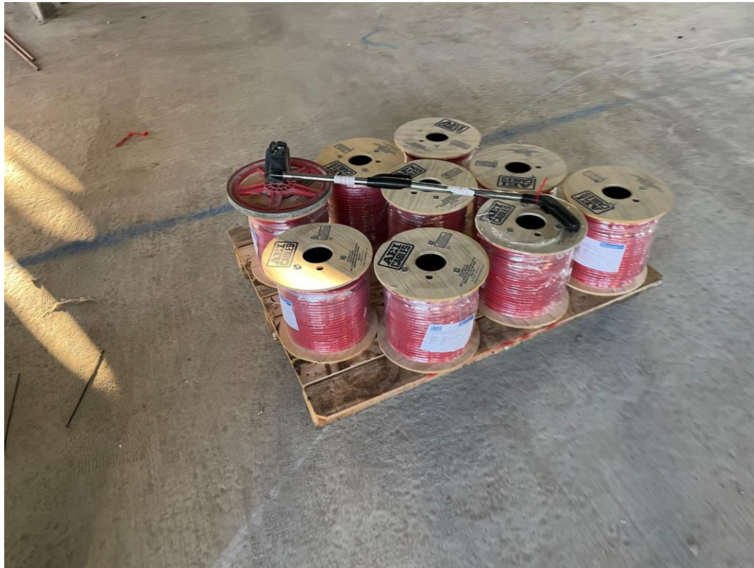
Material Storage – Electrical cabling
