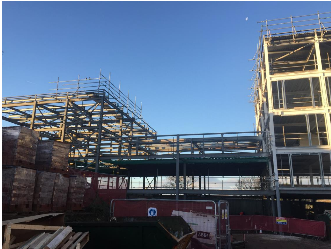
Steel frame structure – Commercial block
