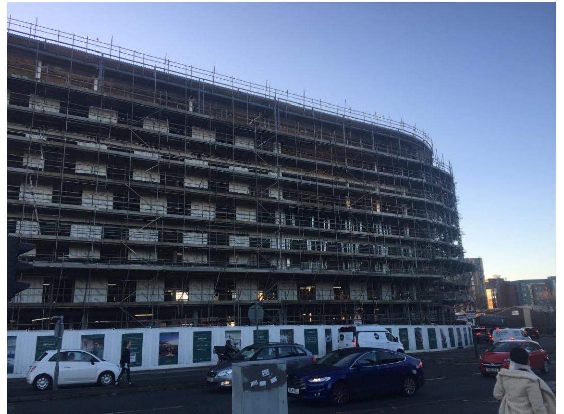
West Derby Road - Site view
