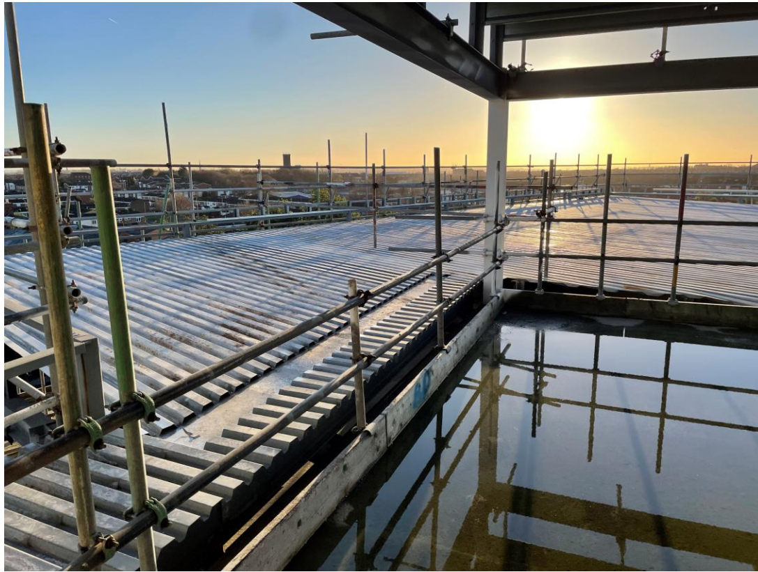
Metal decking structure to roof – Student wing
