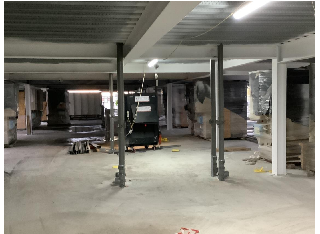
Above ground drainage installation on going to upper floors
