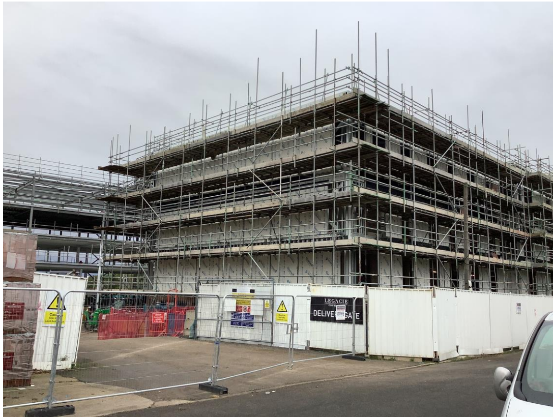
Walker Street - Site view
