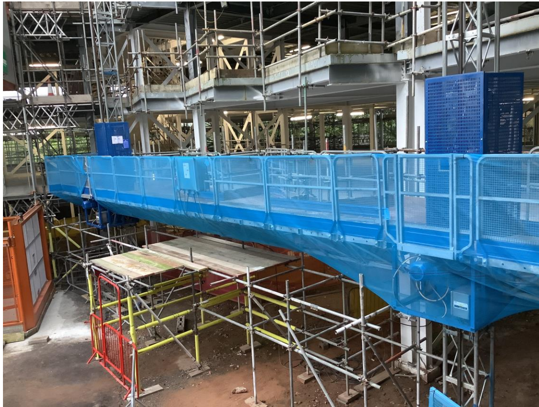
Mast climber installation complete to 'Zig-Zag' Elevation
