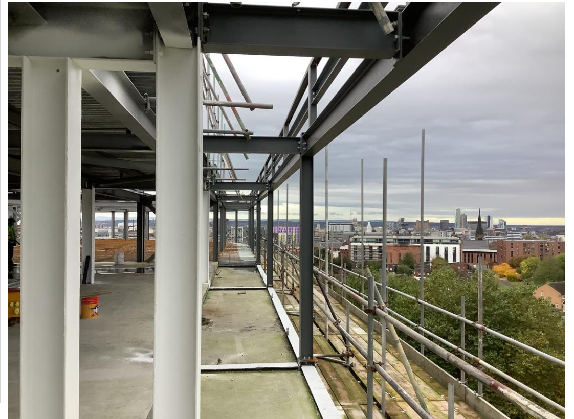
Steel frame modifications and balcony removal works on going
