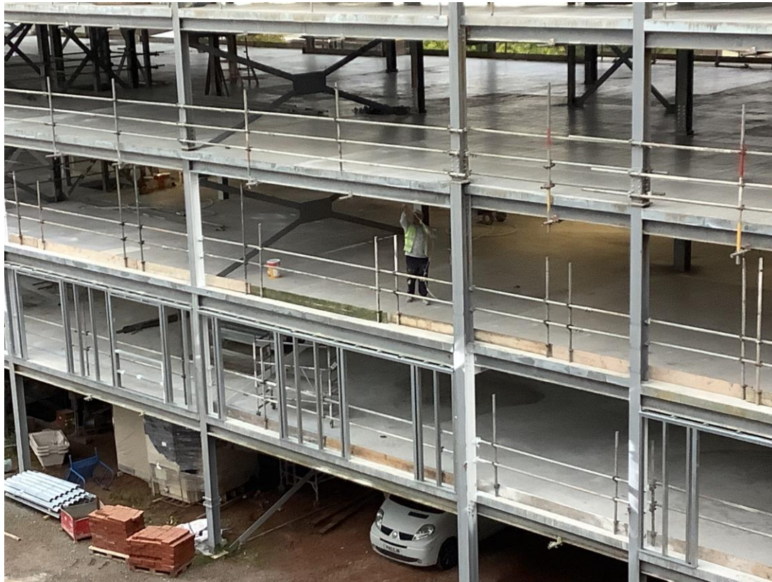
Residential wing – Fire protective coatings on going
