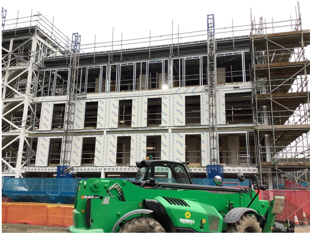
Site access plant
