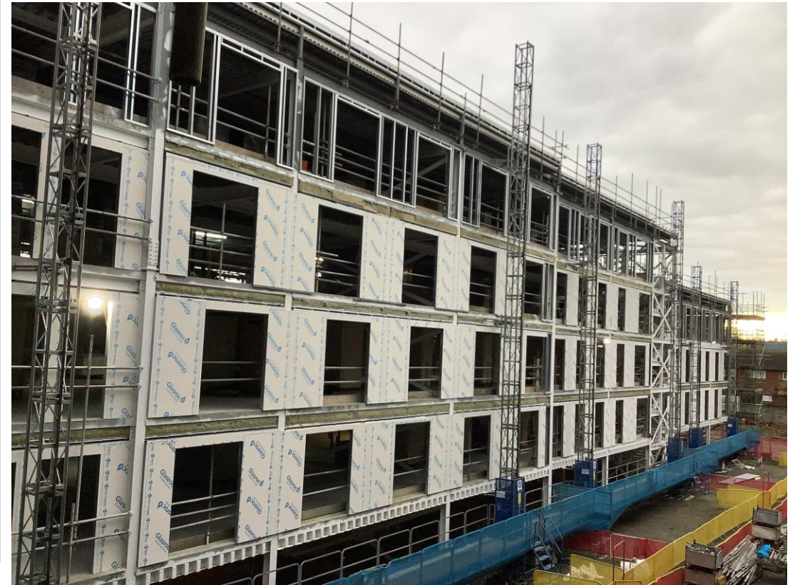
External SFS & sheathing board installation ongoing
