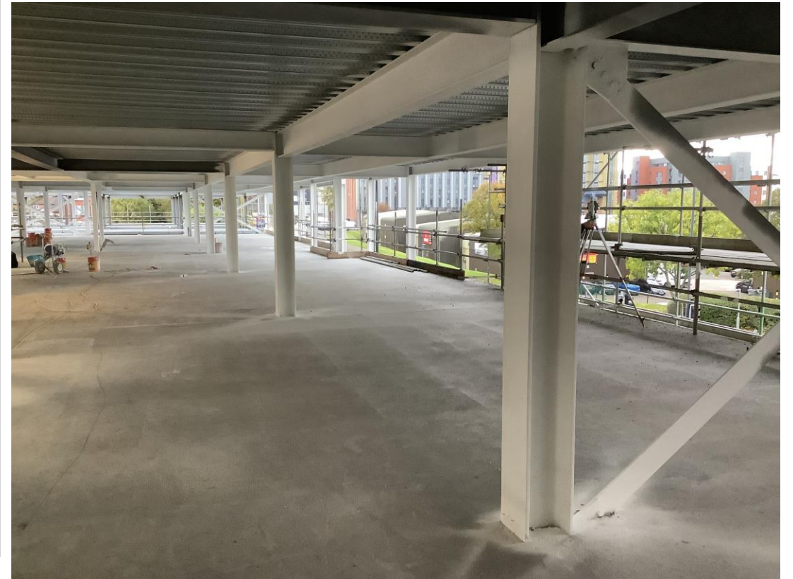
Residential wing – Fire protective coatings on going
