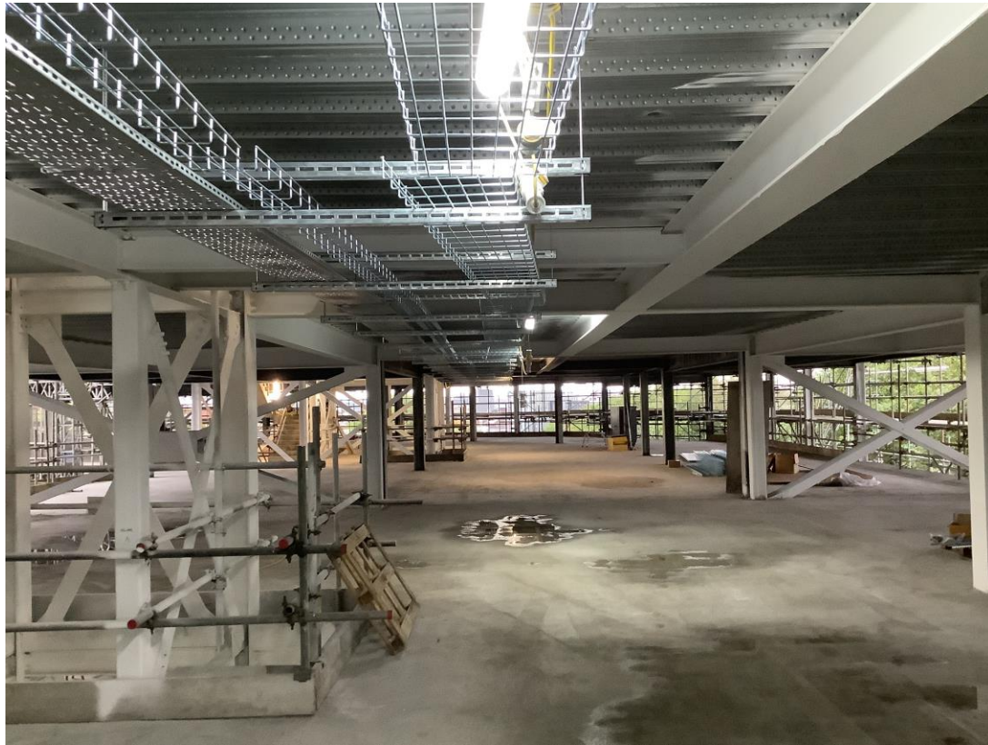
Electrical containment installation on going to student wing
