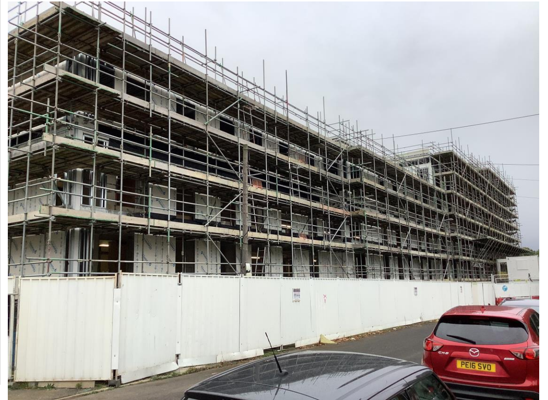
Walker Street - Site view
