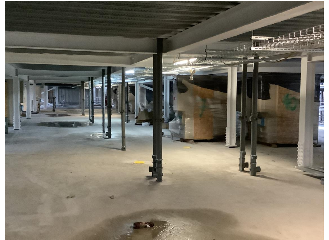
Above ground drainage installation on going
