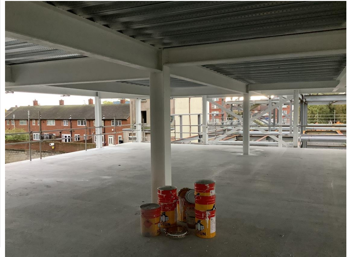
Residential wing – Fire protective coatings on going
