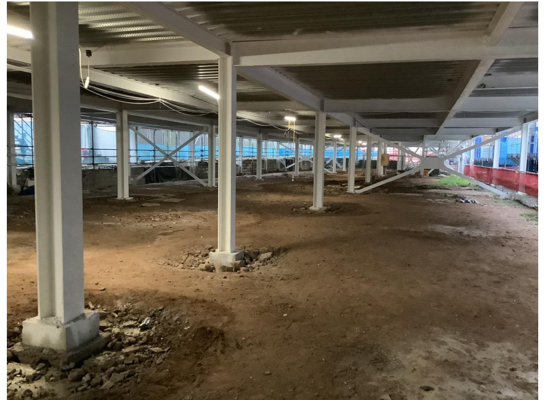
Undercroft Parking Area
