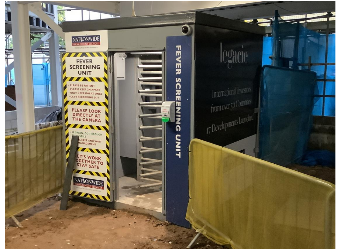
Site access barriers and turnstile being utilised
