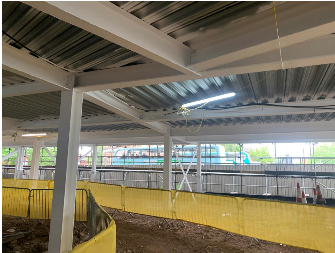
Site access barriers installed
