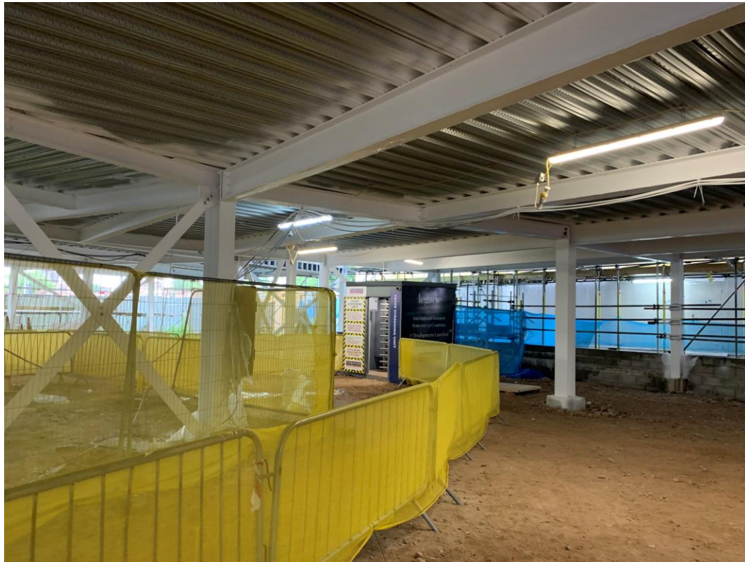
Site access barriers and turnstile being utilised
