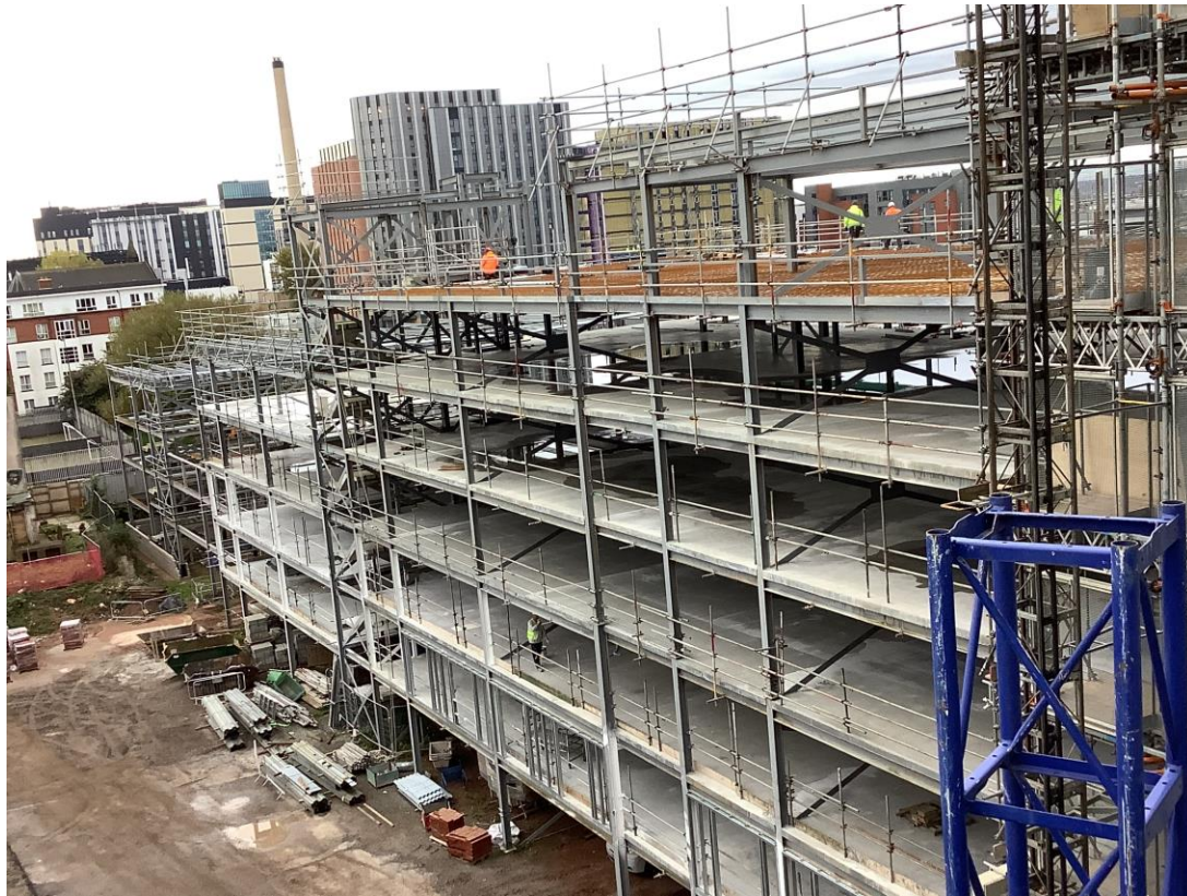
Concrete floor slab – Concrete slab pours nearing completion to Residential wing
