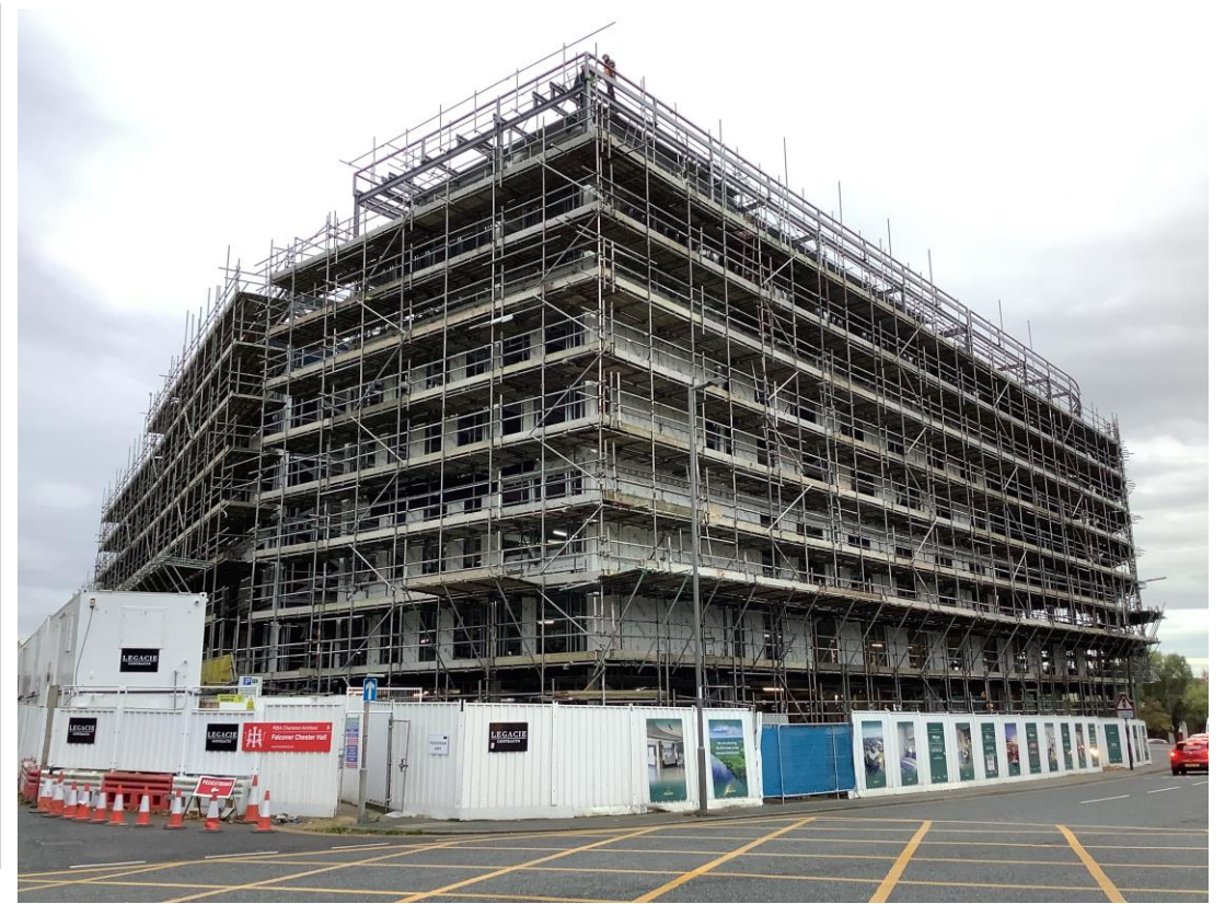
West Derby Road - Site view
