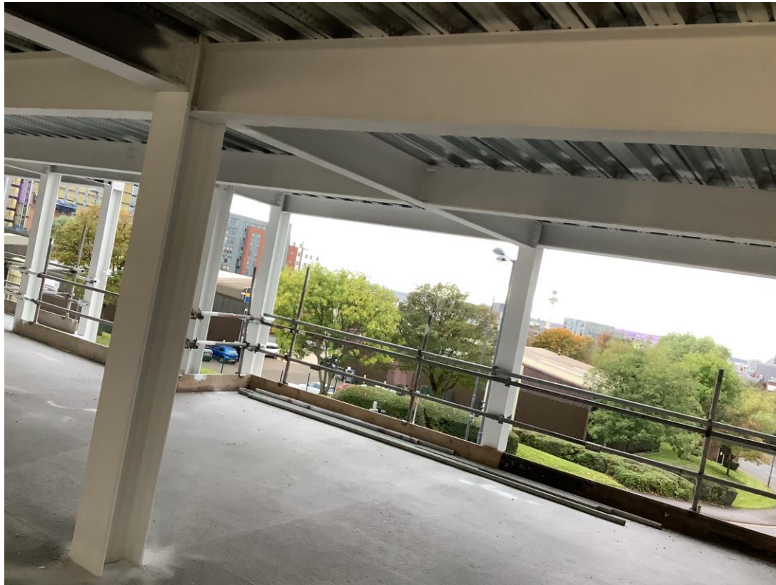
Residential wing – Fire protective coatings on going
