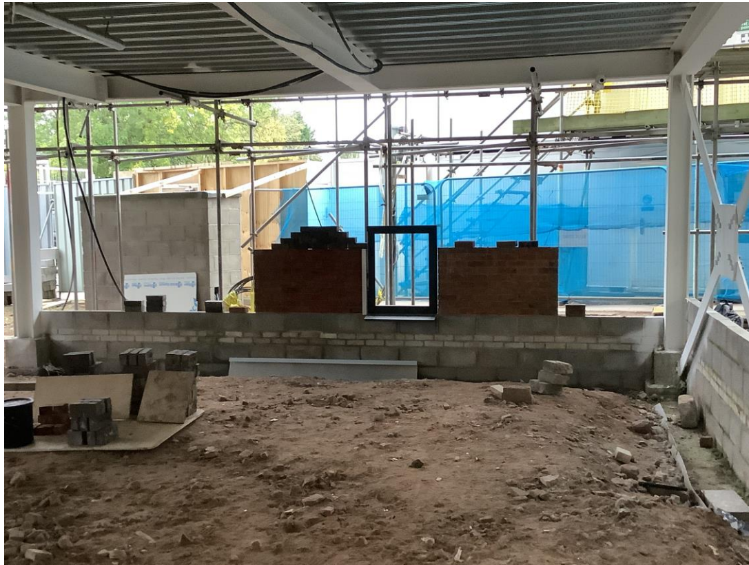
Brickwork Mock Up
