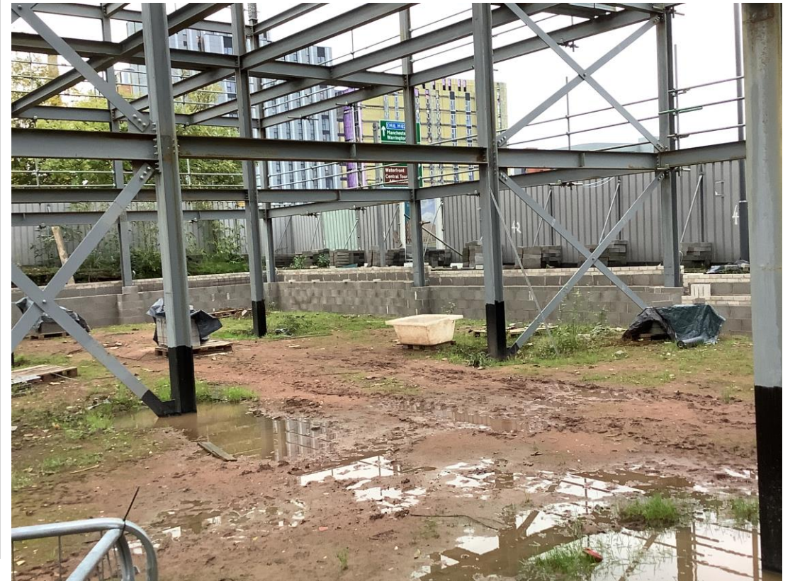
Construction of new retaining wall structure on going
