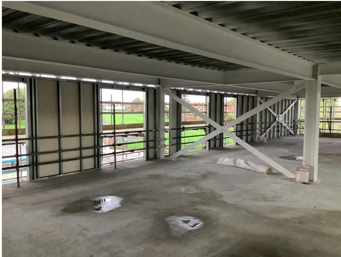
External SFS & sheathing board installation ongoing
