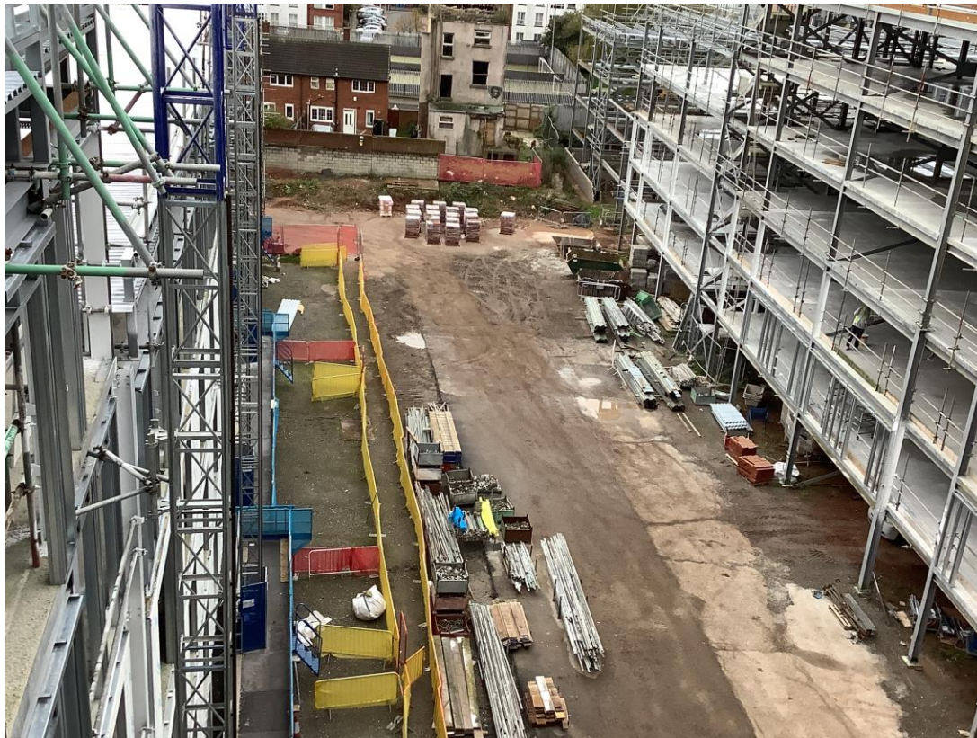
Inner courtyard view, steel framework structure
