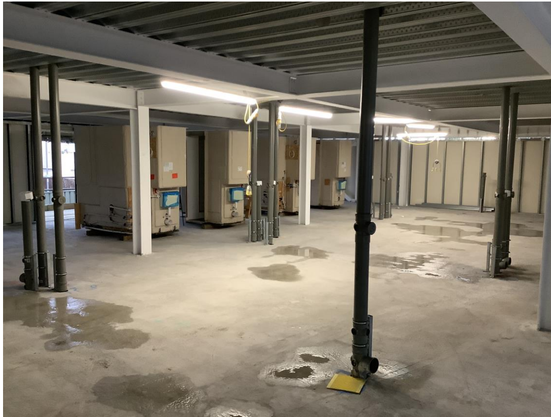
Above ground drainage installation on going
