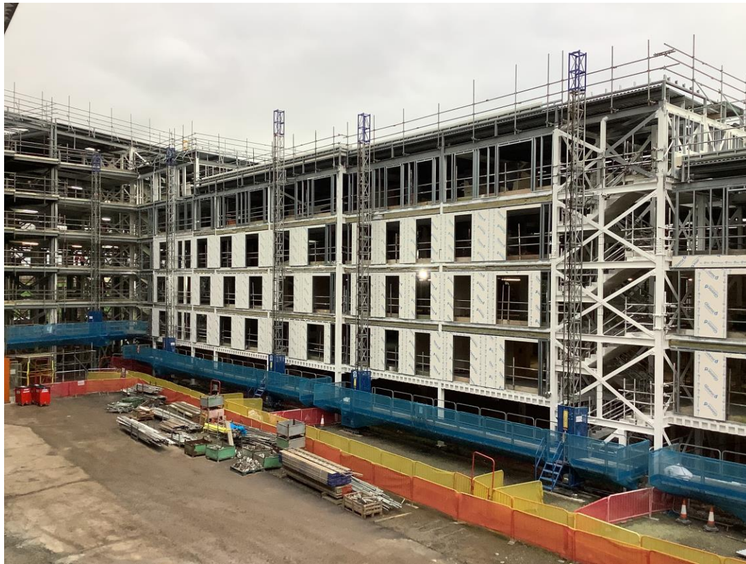
Inner courtyard view, steel framework structure, SFS & mast climbers
