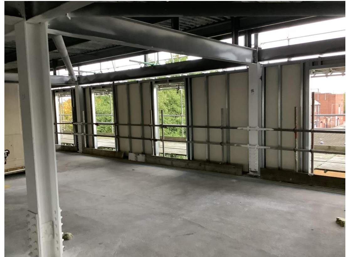
External SFS & sheathing board installation ongoing
