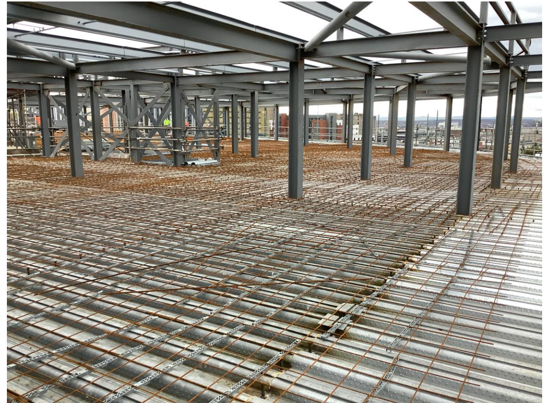
Steel framework structure to upper floors – Concrete pouring due to commence
