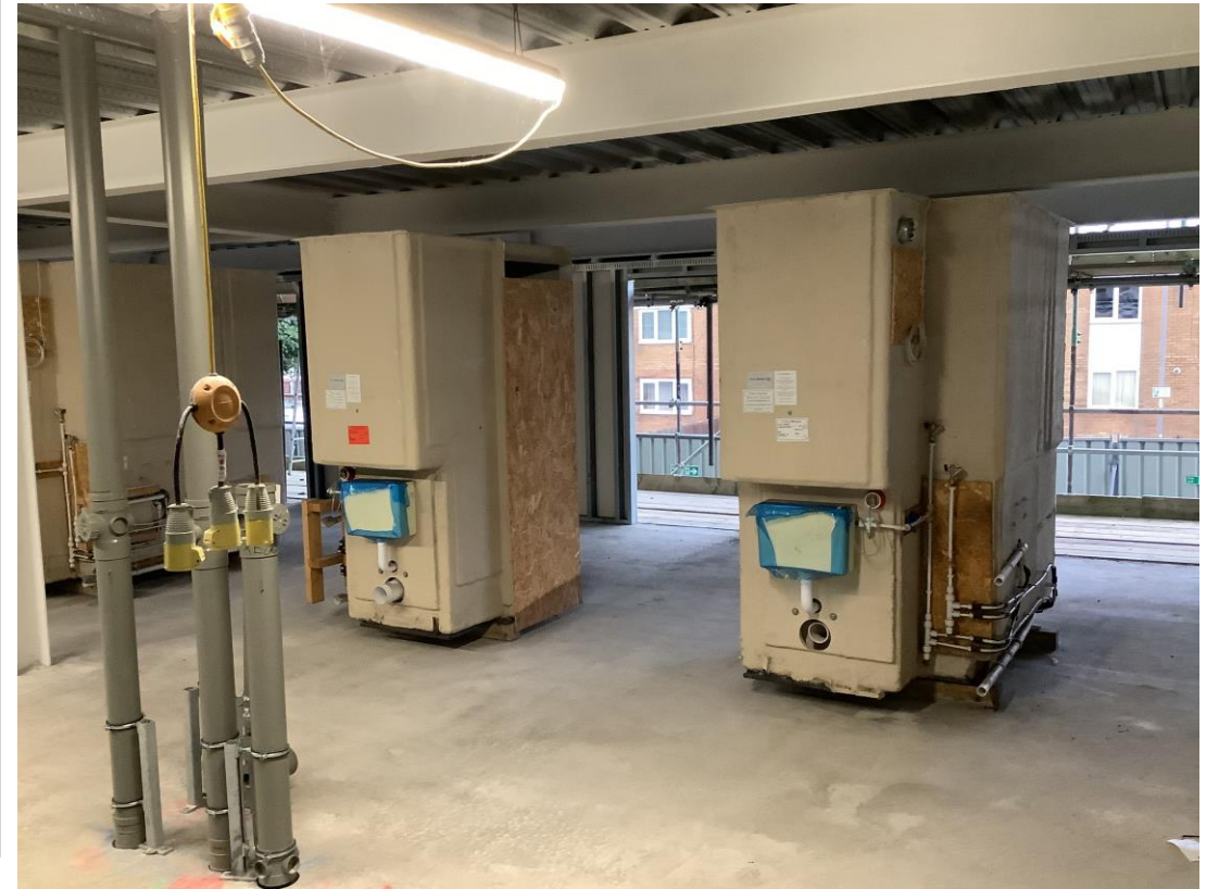
Bathroom pod testing and itinerary checks complete in preparation for installation
