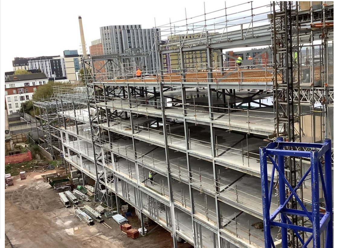
Steel framework structure
