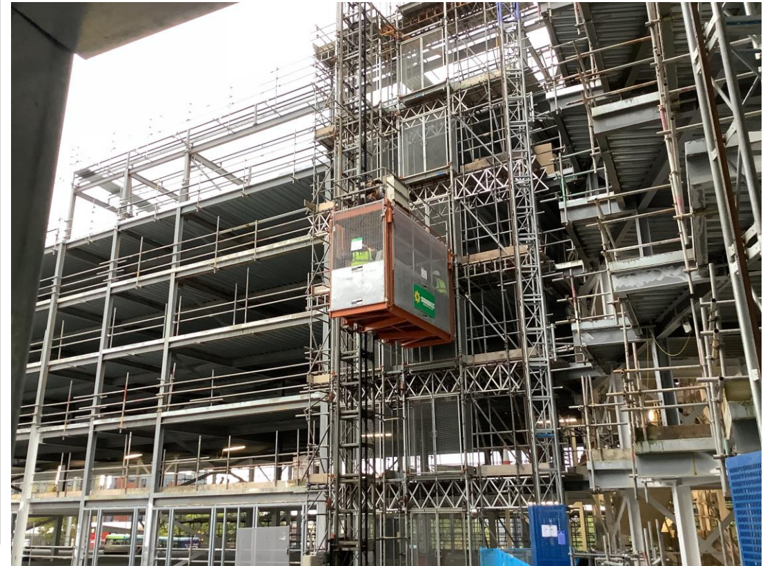
Installation of temporary construction elevator complete
