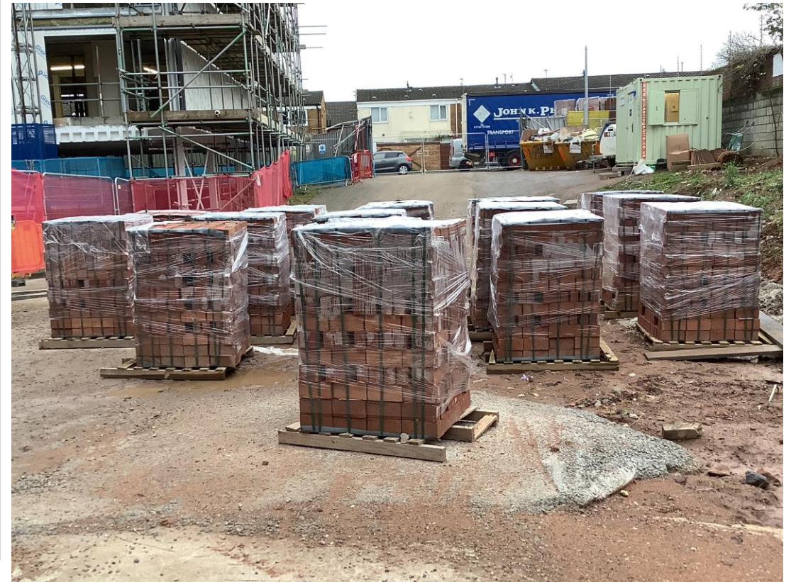
Material storage – Red Brick
