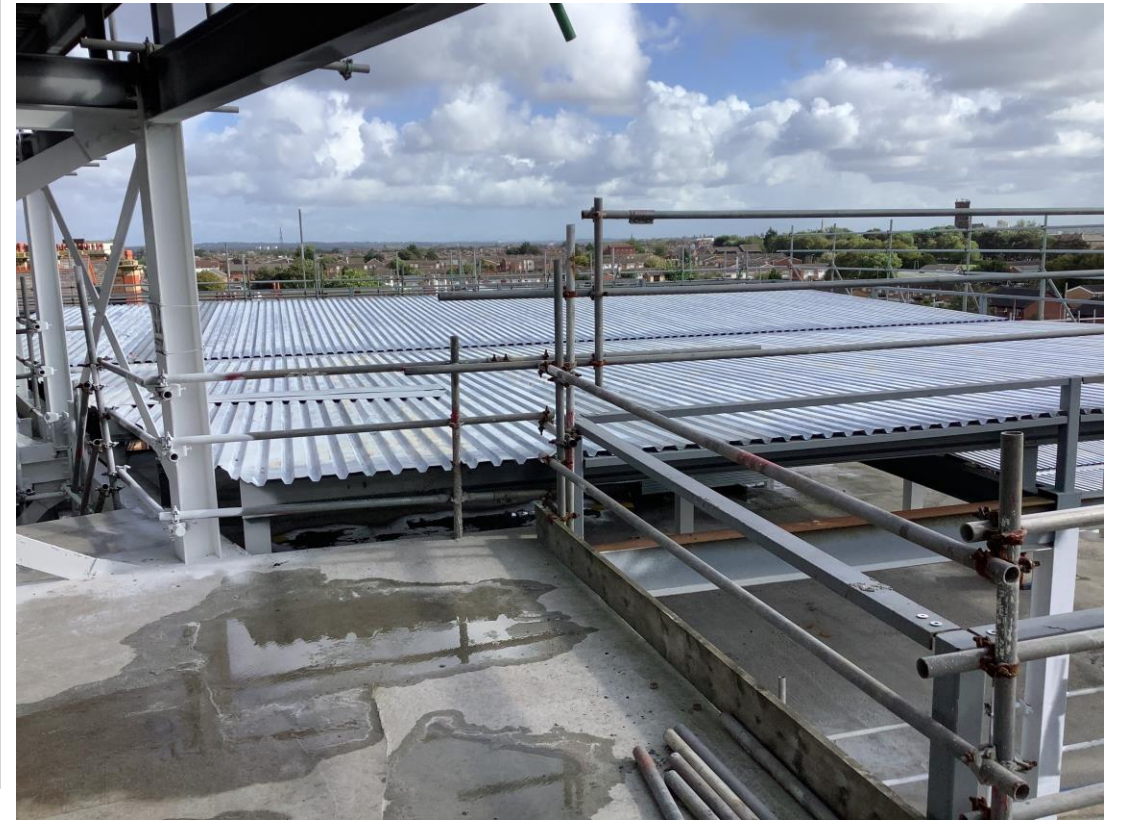
Metal decking structure to upper floors
