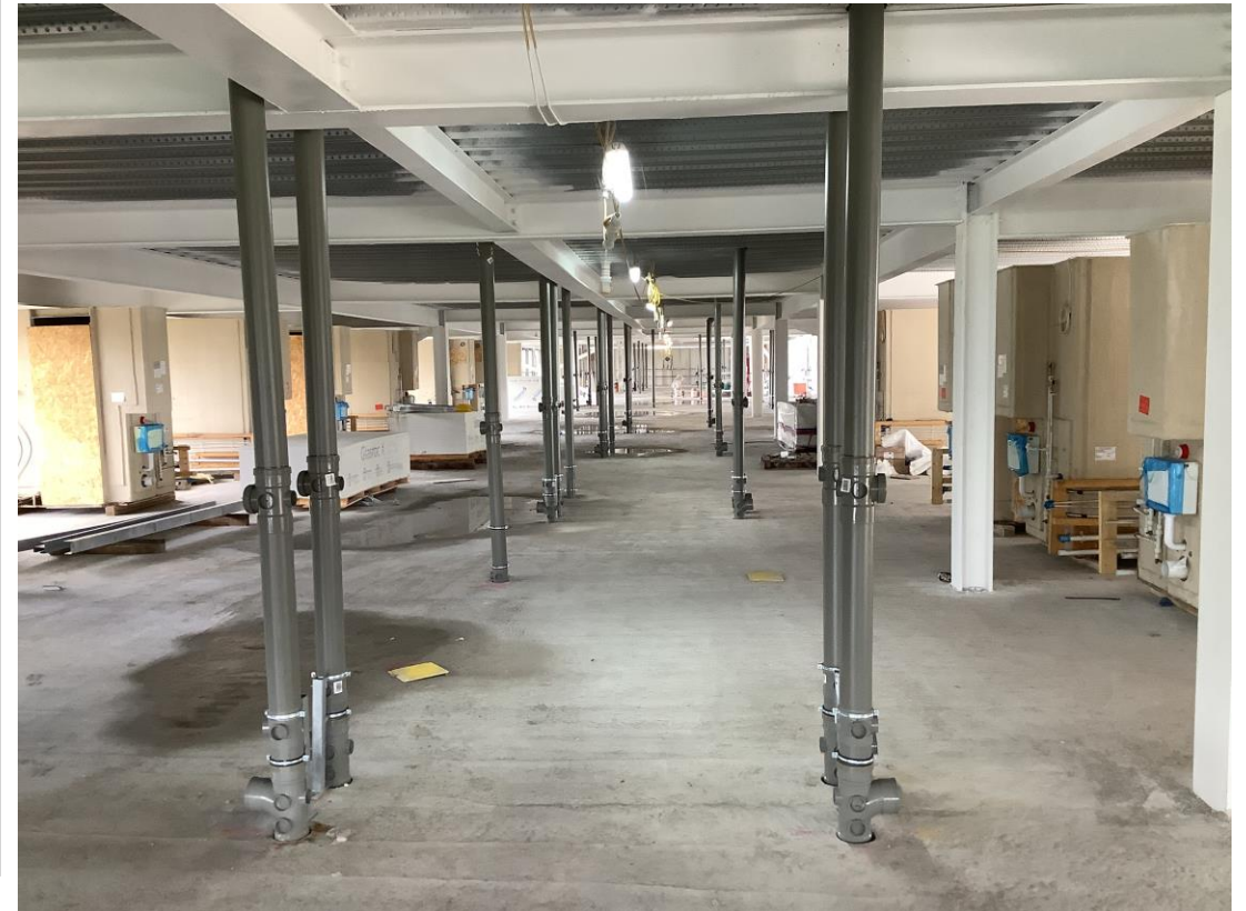
Above ground drainage installation on going to second floor
