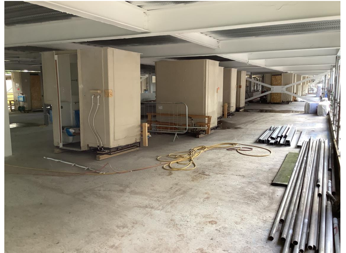
Pod testing and itinerary checks complete ready for installation
