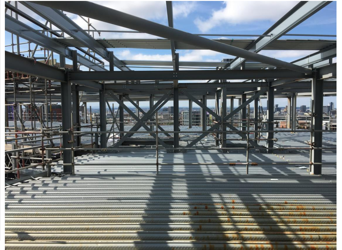
Steel framework structure to upper floors
