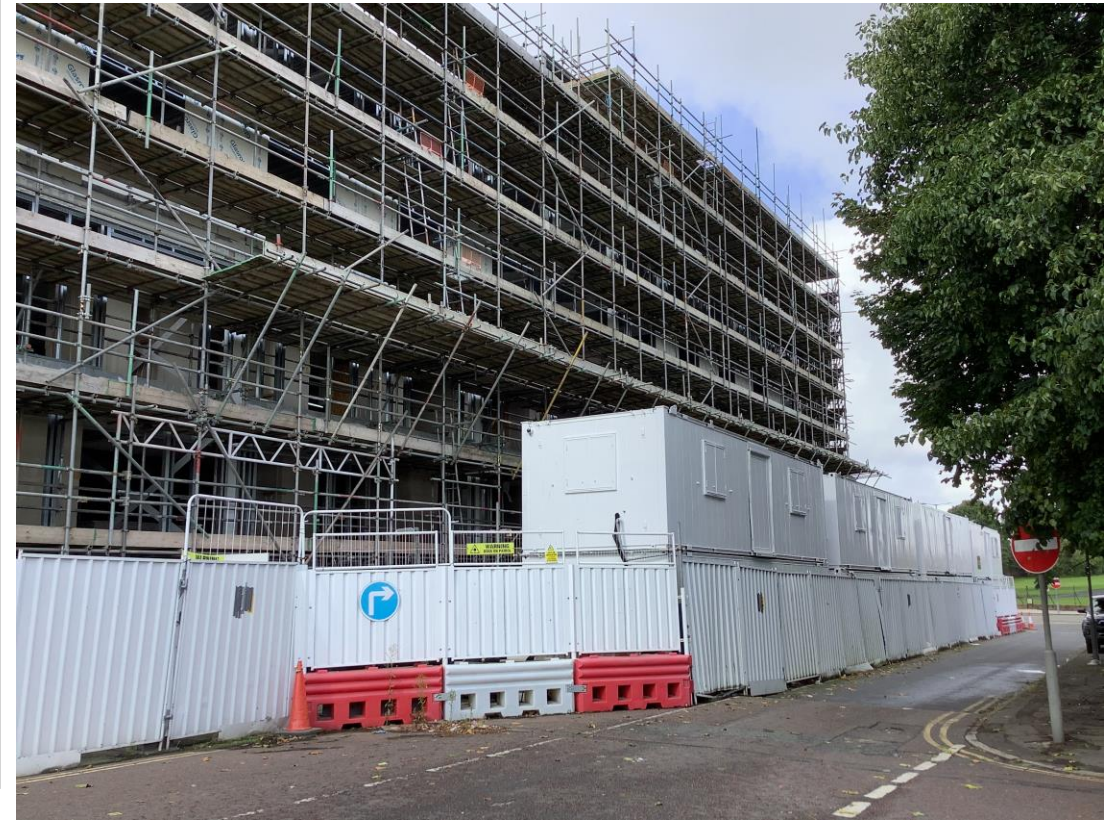
Walker Street - Site view
