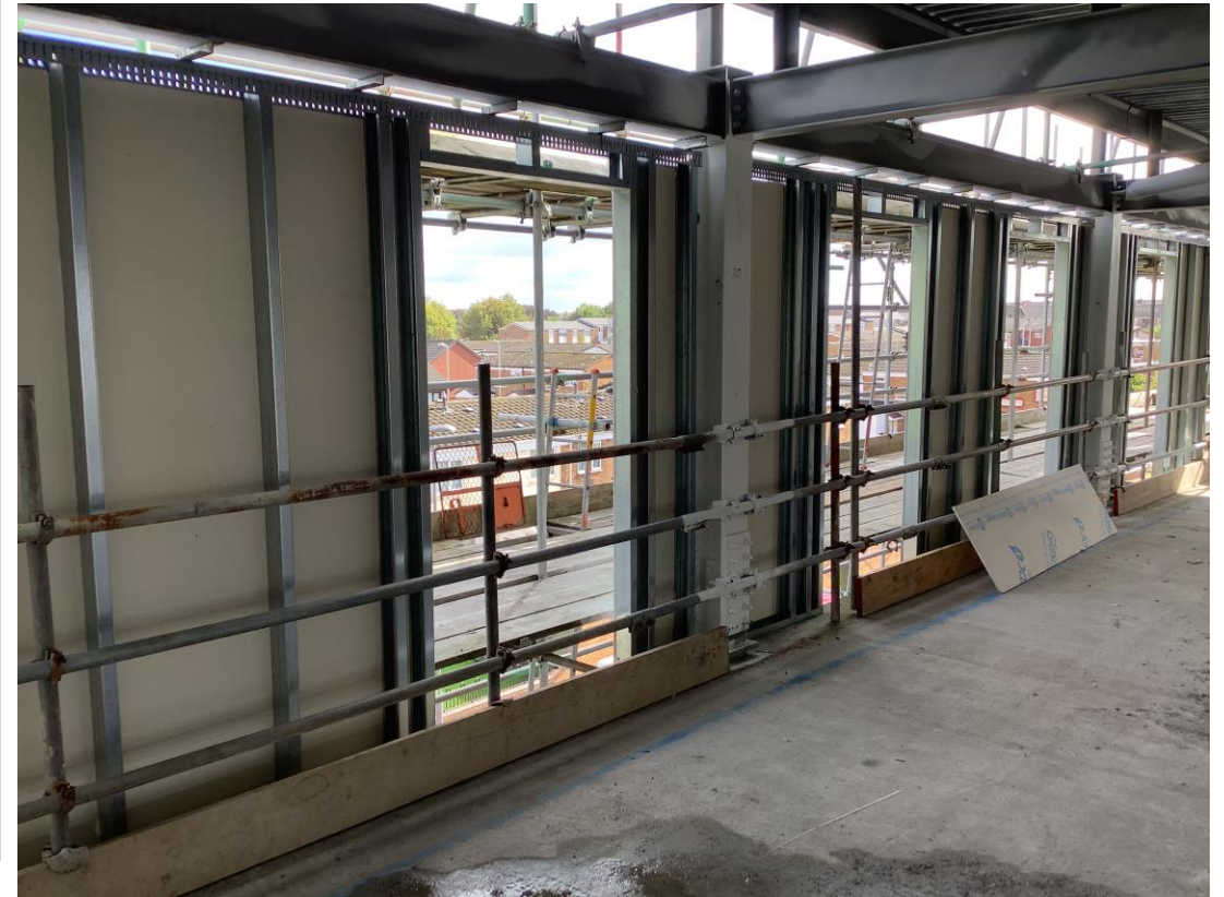
External sheathing board installation ongoing
