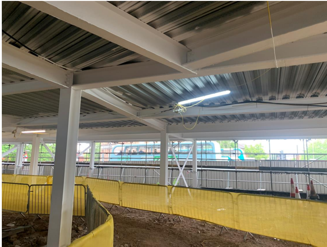
Site access barriers installed
