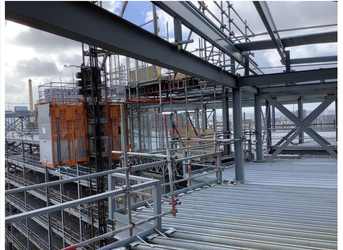
Steel framework structure & industrial elevator
