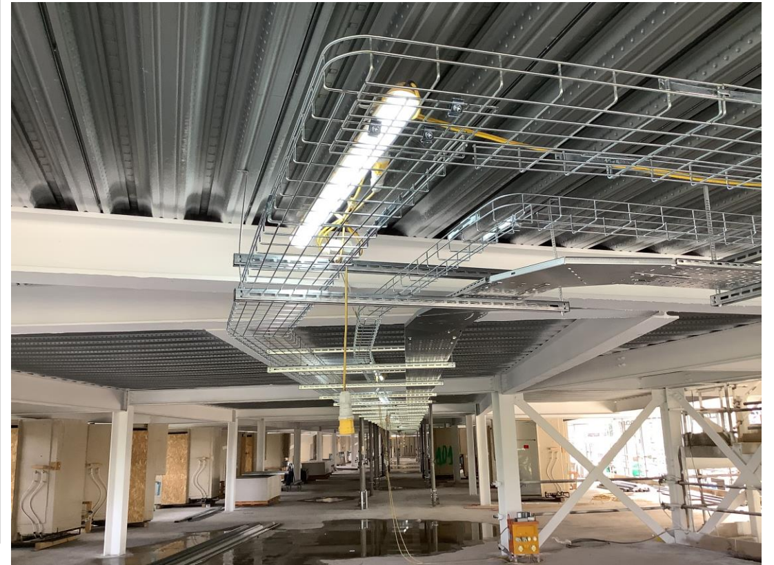
Electrical containment installation commenced to first floor
