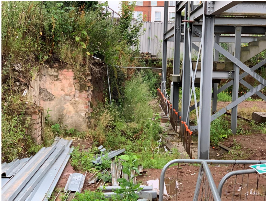
New retaining wall structure commenced
