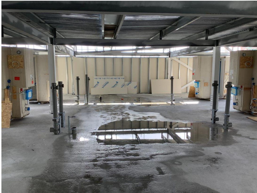
External sheathing board installation ongoing
