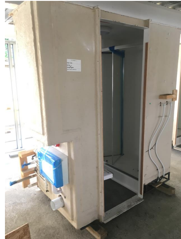
Bathroom pods delivered for installation – Pod testing and itinerary checks complete
