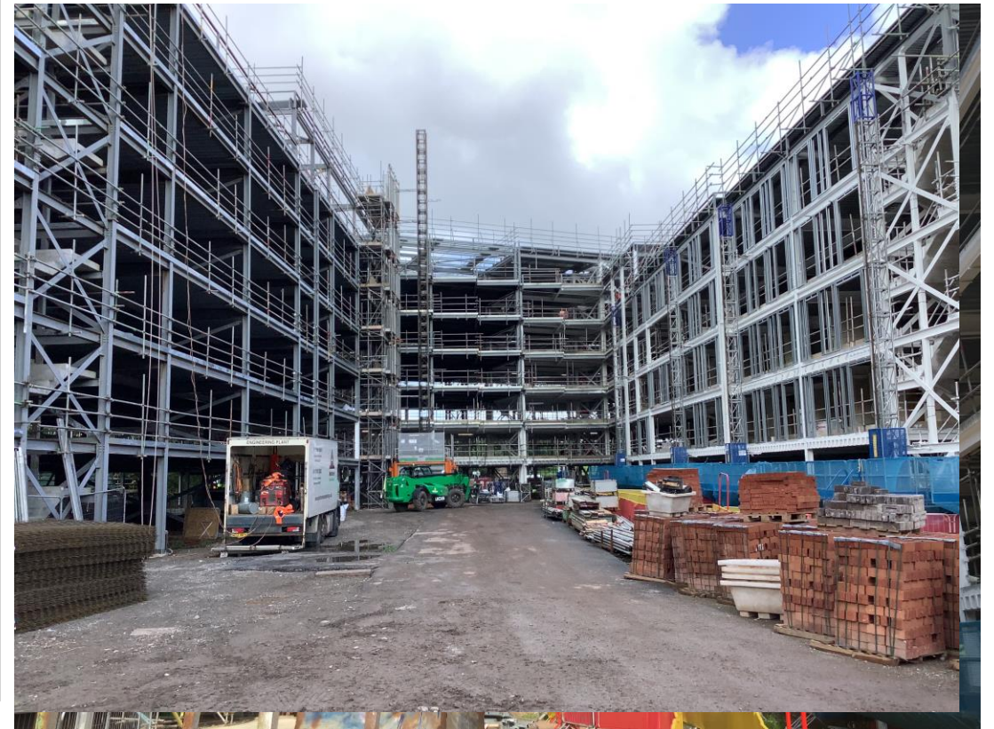
Inner courtyard view steel framework structure
