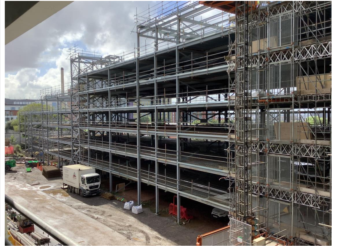
Inner courtyard area
