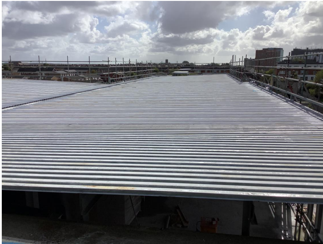
Metal decking structure to upper floors
