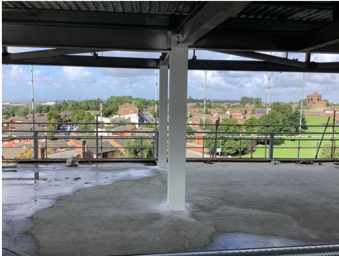
Steel framework structure upper floors – Fire protective coatings ongoing
