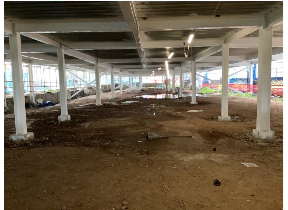
Undercroft Parking Area
