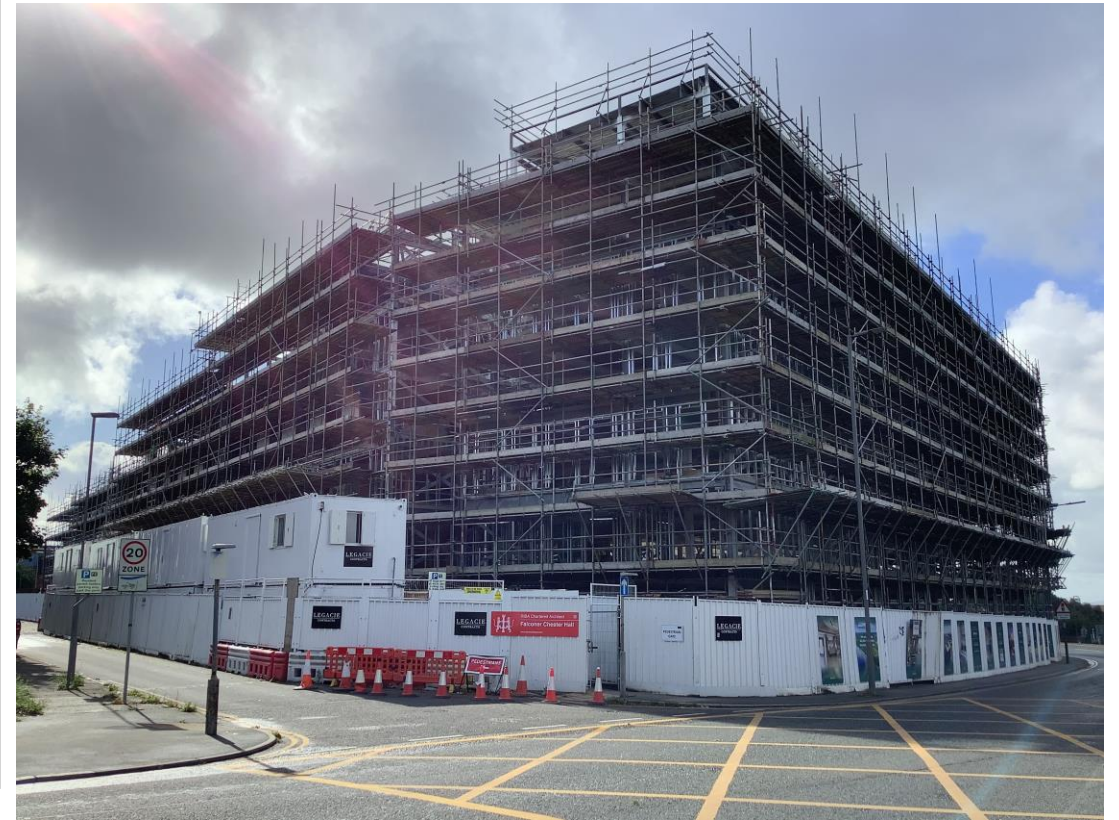
West Derby Road - Site view
