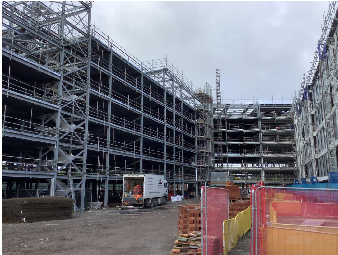
Courtyard scaffold – Scaffold safety checks complete
