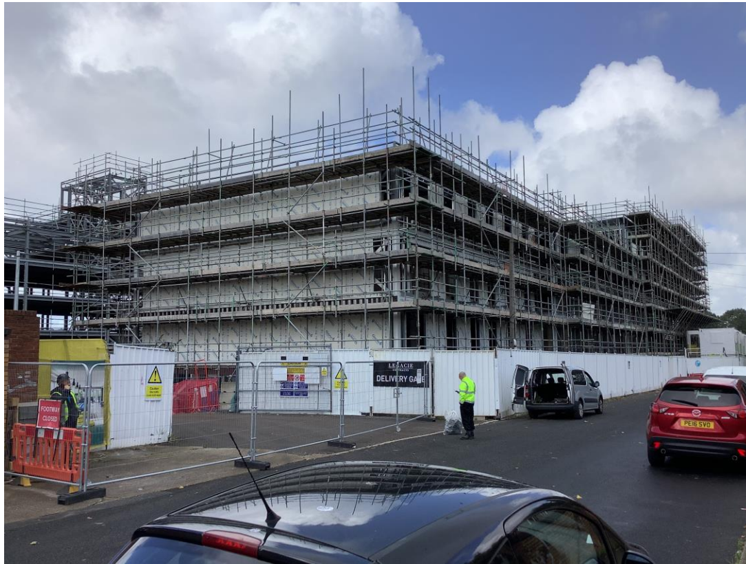
Walker Street - Site view
