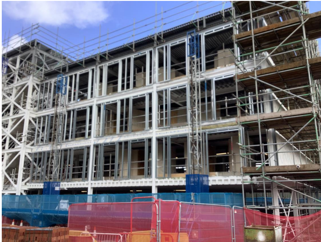
Steel framework structure and SFS on going
