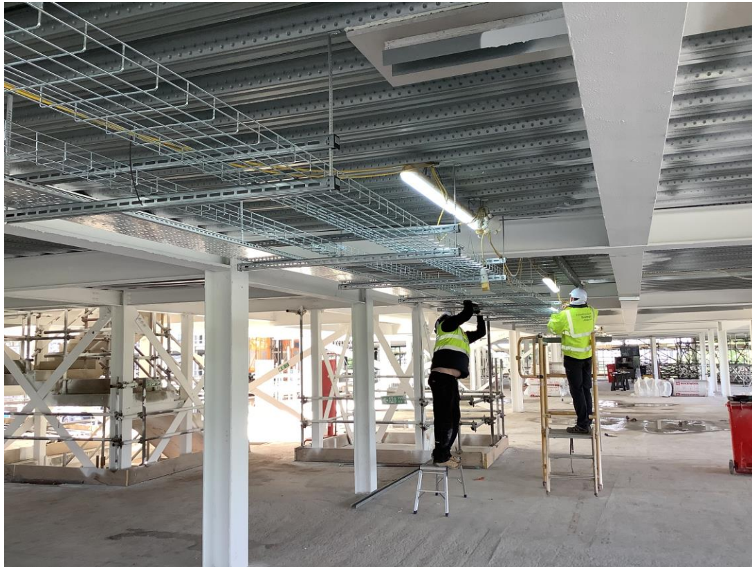
Electrical containment installation commenced to first floor
