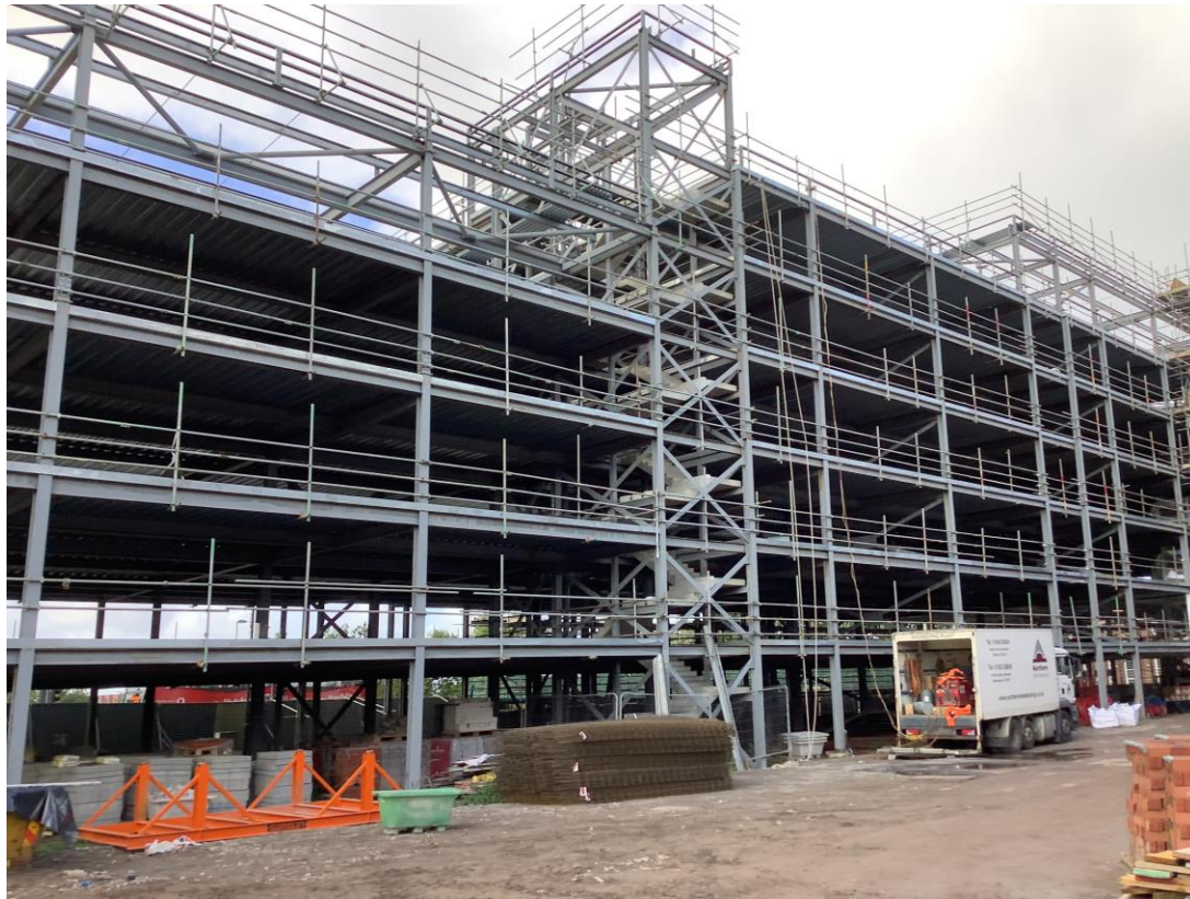
Inner courtyard view steel framework structure & stair core
