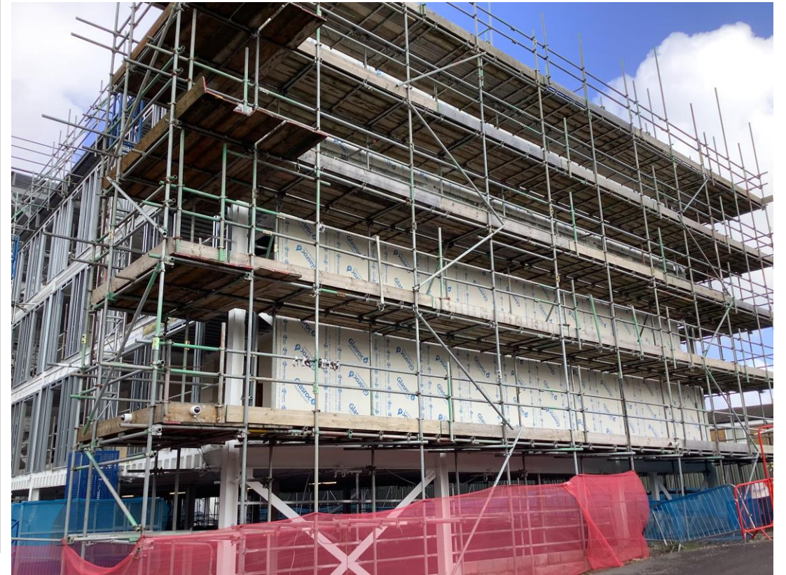
Steel framework structure and external sheathing board installation on going
