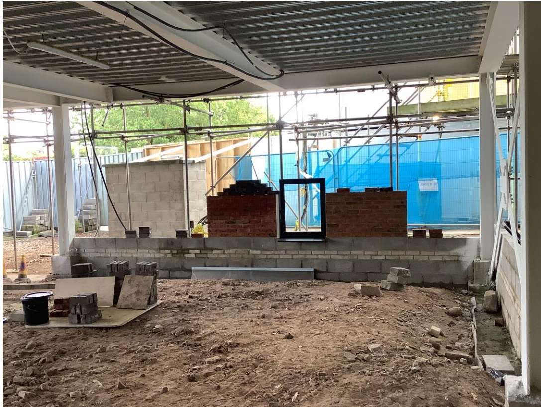
Brickwork Mock Up
