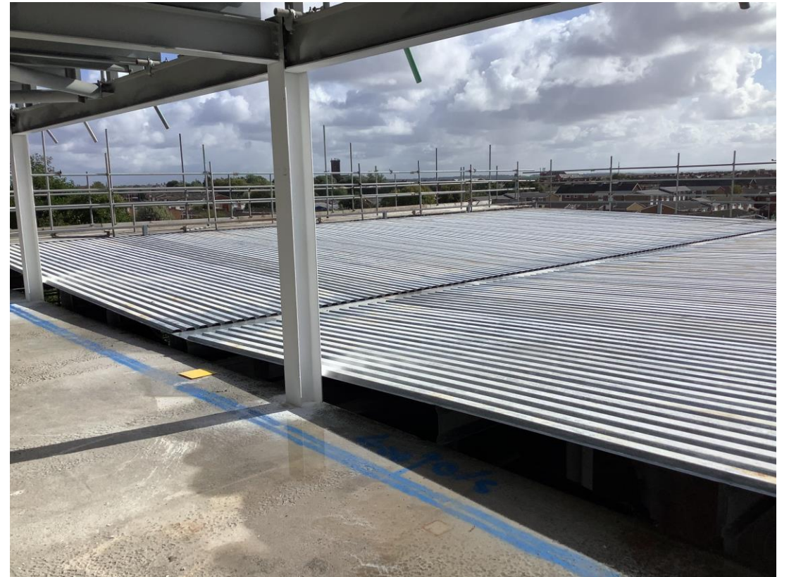
Metal decking structure to upper floors
