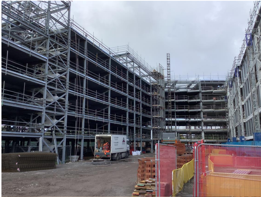
Inner courtyard area
