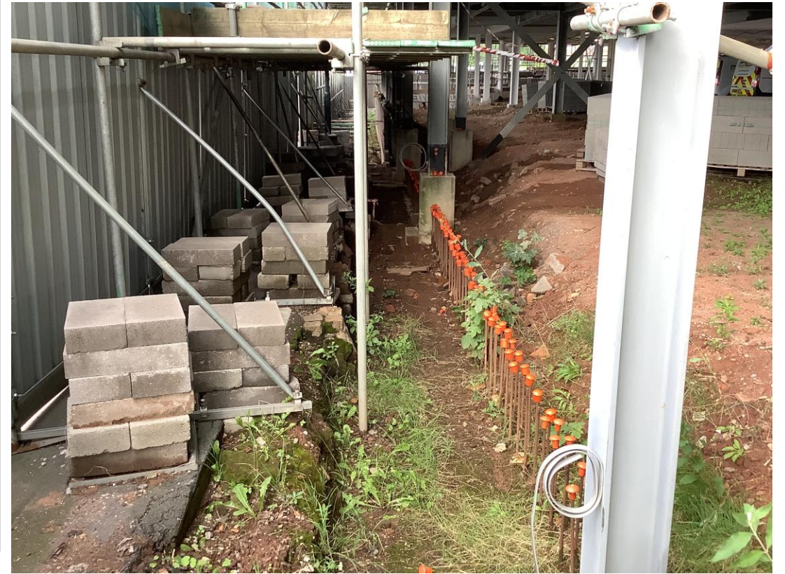
New retaining wall structure commenced
