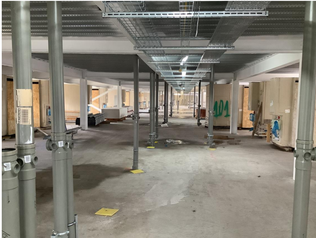
Electrical containment installation commenced to first floor
