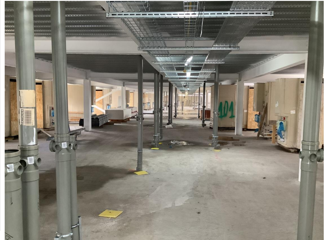
Above ground drainage installation on going to first floor
