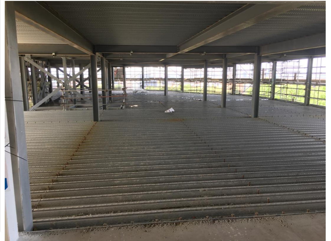
Metal decking structure to lower floors – Concrete pouring yet to re-commence
