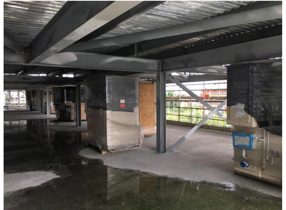
Steel framework structure to upper floors – Fire protective coatings commenced
