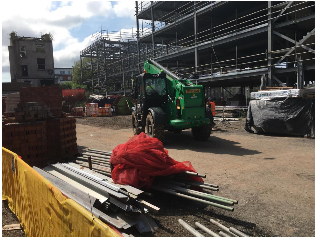
Material storage and site access plant
