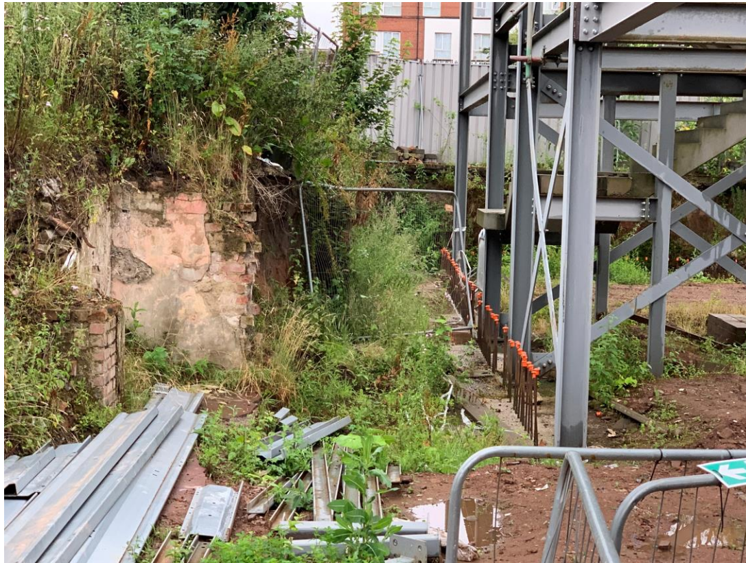
New retaining wall structure commenced
