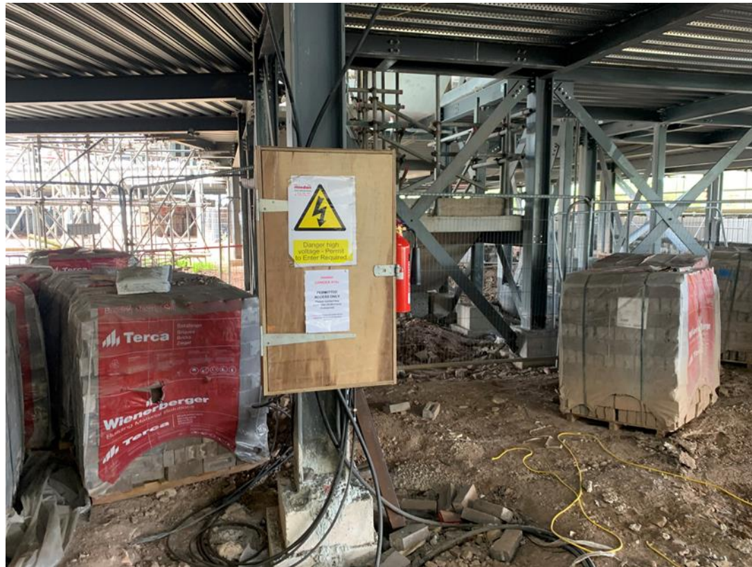
Electrical supply installed
