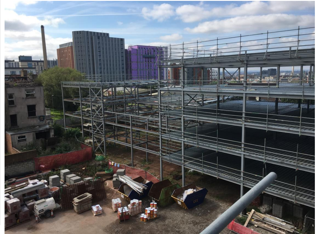
Steel frame structure and metal decking ongoing
