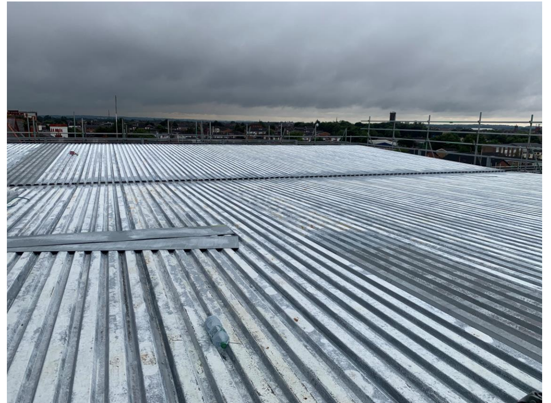
Metal deck roof structure
