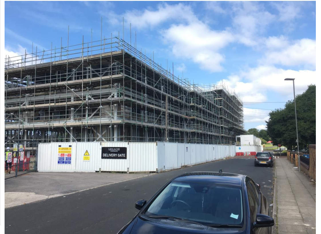
Walker Street - Site view
