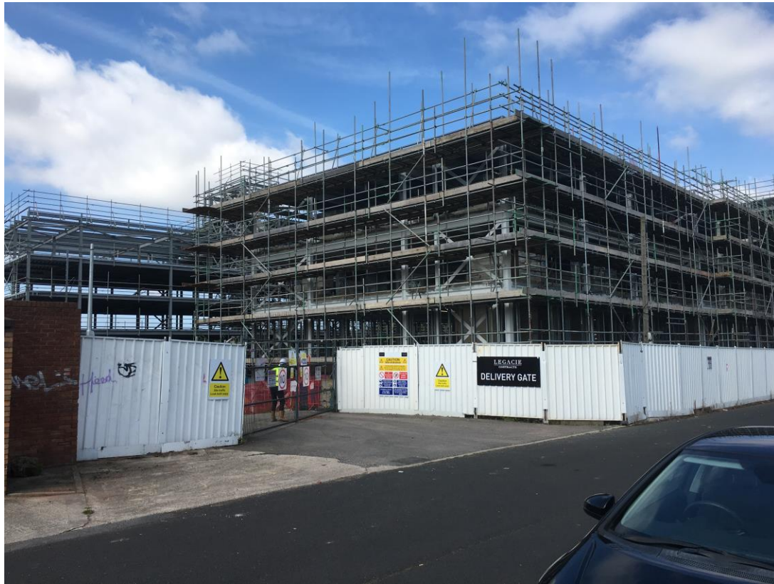
Walker Street - Site view
