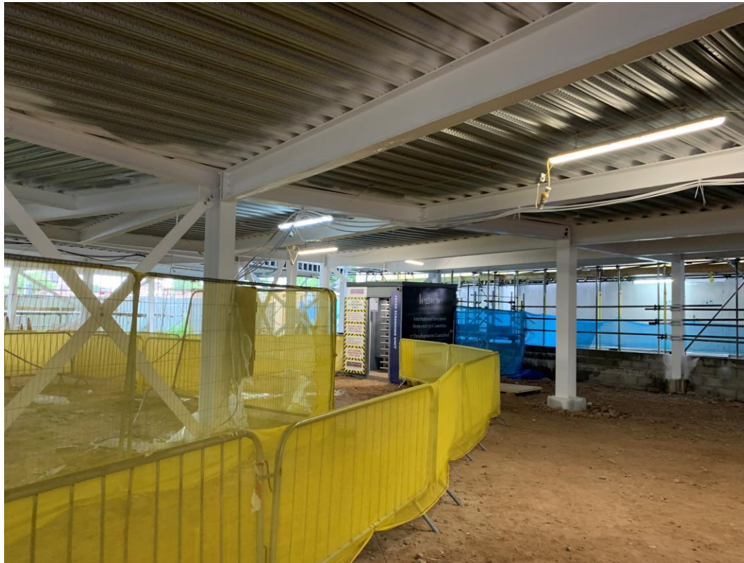
Site access barriers and turnstile installed
