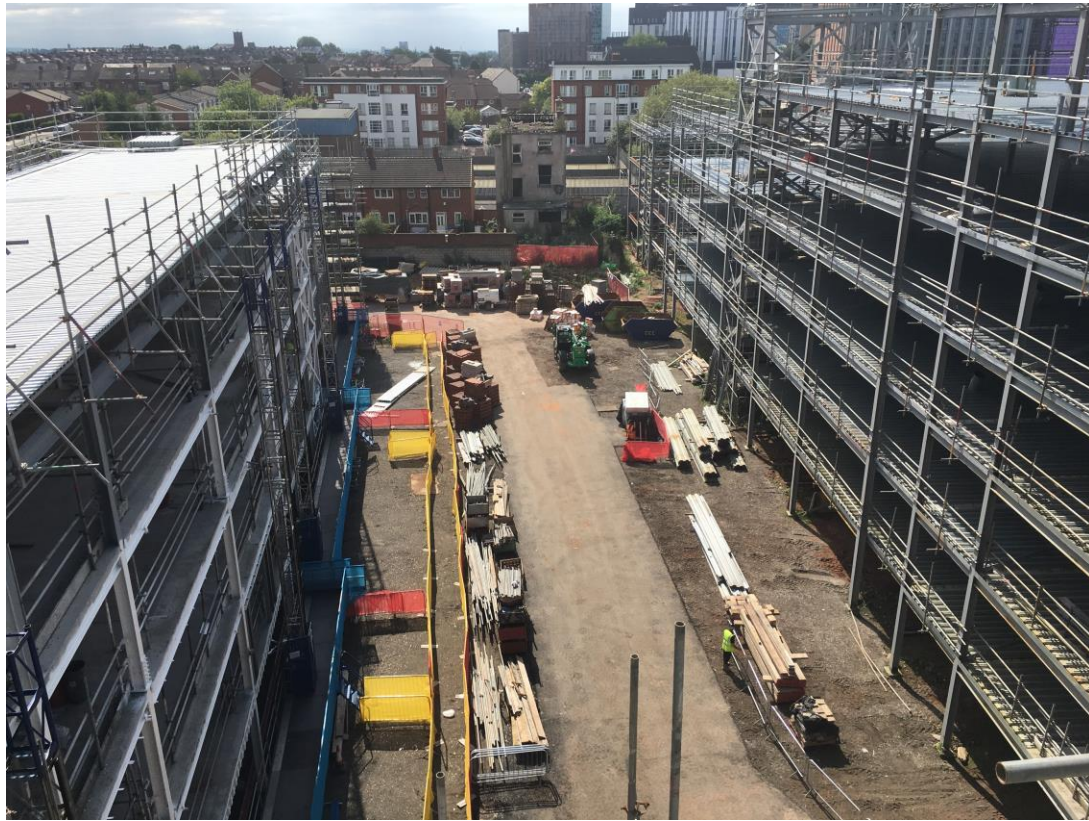
Aerial view of the courtyard, site storage and access road
