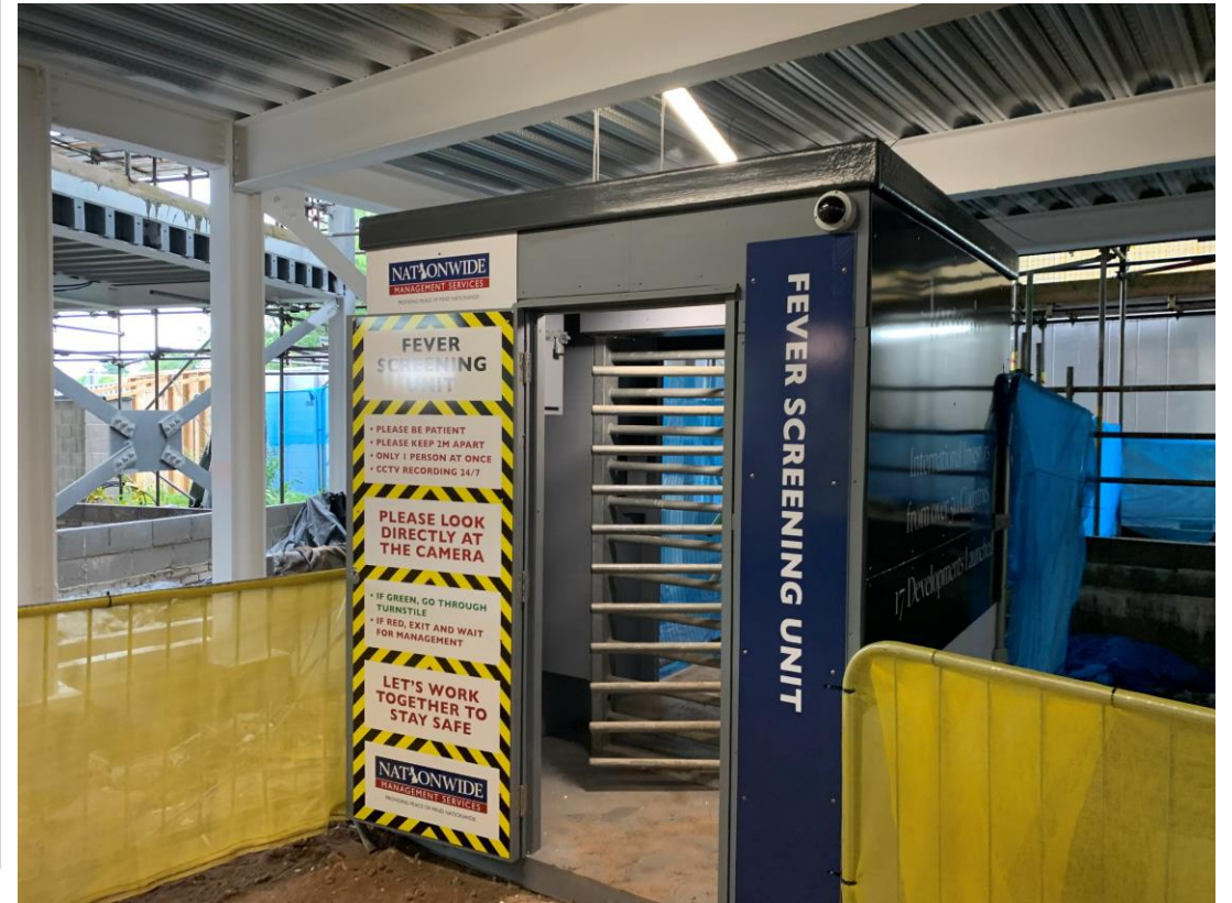
Site access barriers and turnstile installed
