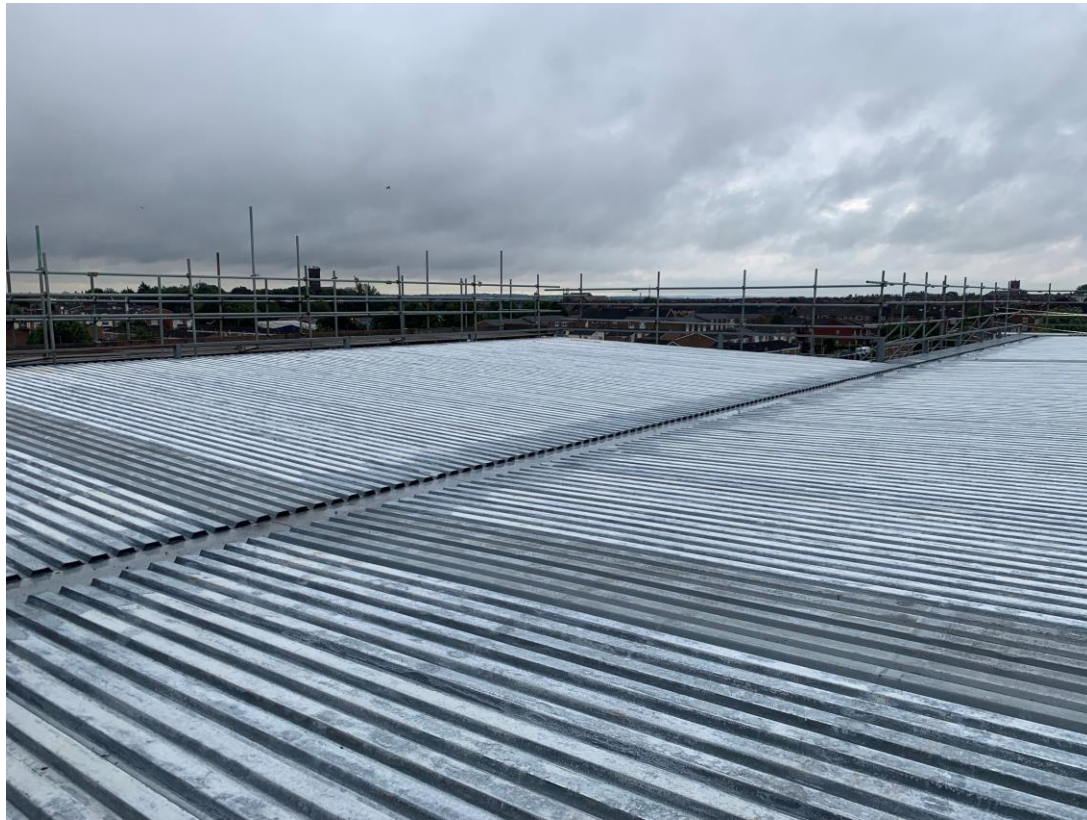
Metal deck roof structure
