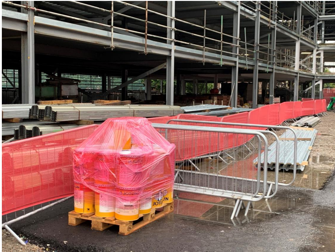
Site materials stored
