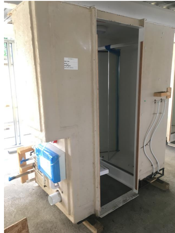
Bathroom pods delivered for installation – Pod testing and itinerary checks currently ongoing
