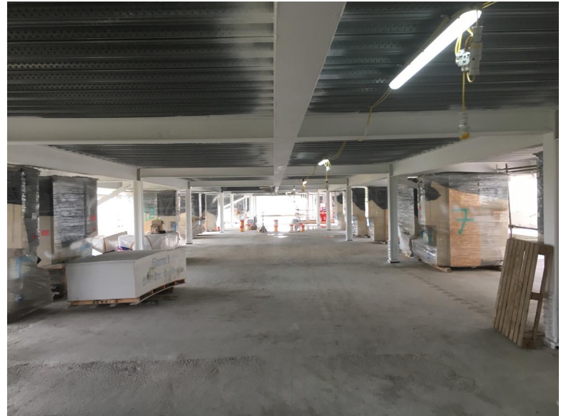
Temporary lighting installation ongoing as required
