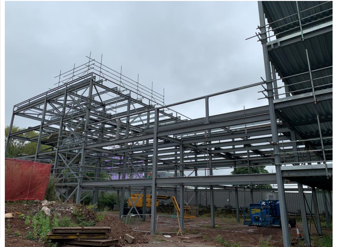
Steel framework structure and decking works ongoing
