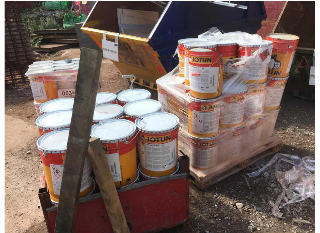
Material Storage – Intumescent paint
