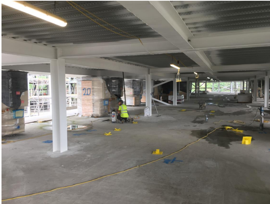
Core drilling ongoing
