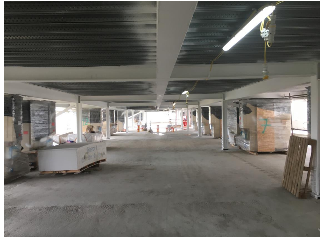
Steel framework structure lower floors – Fire protective coating ongoing
