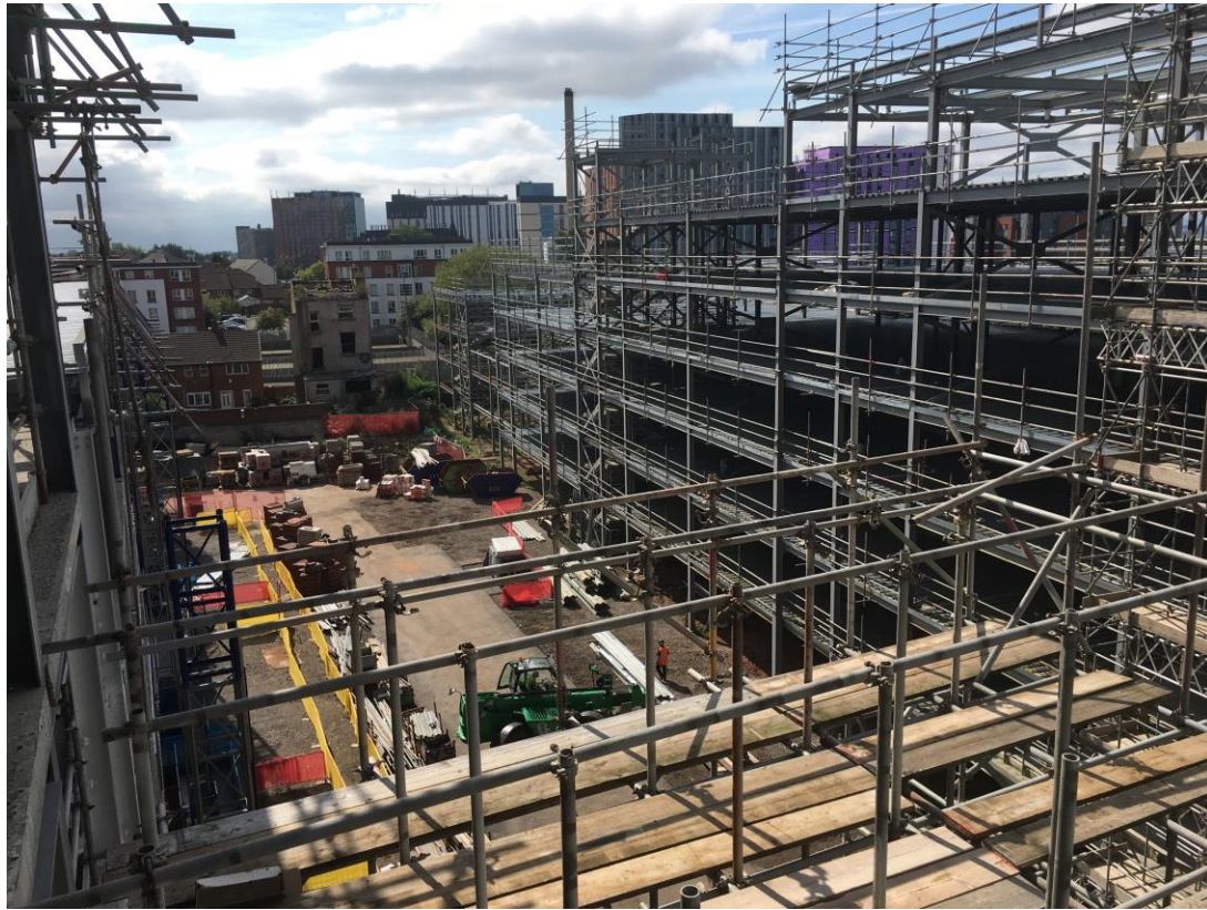
Inner courtyard view steel framework structure & scaffolding
