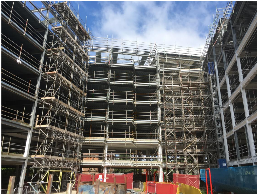
Courtyard scaffold – Scaffold safety checks currently ongoing
