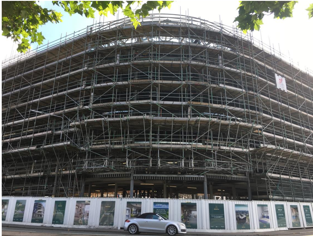
Brunswick Road - Site view
