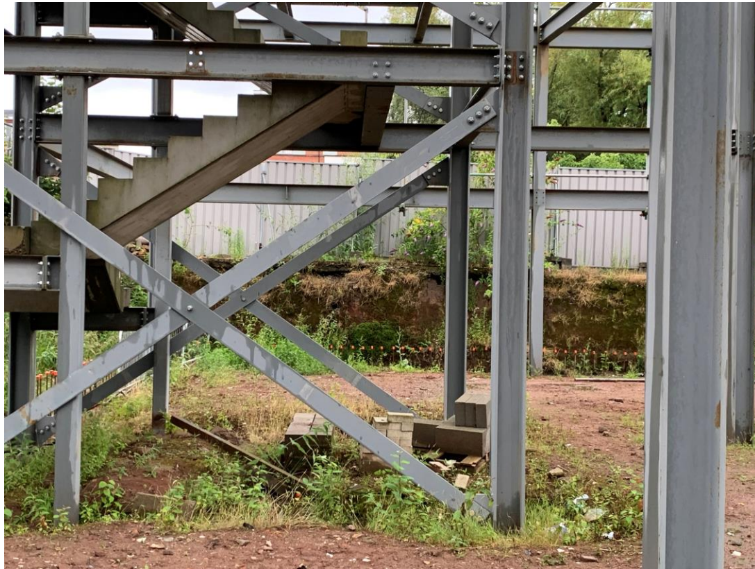
Steel framework and foundation modifications
