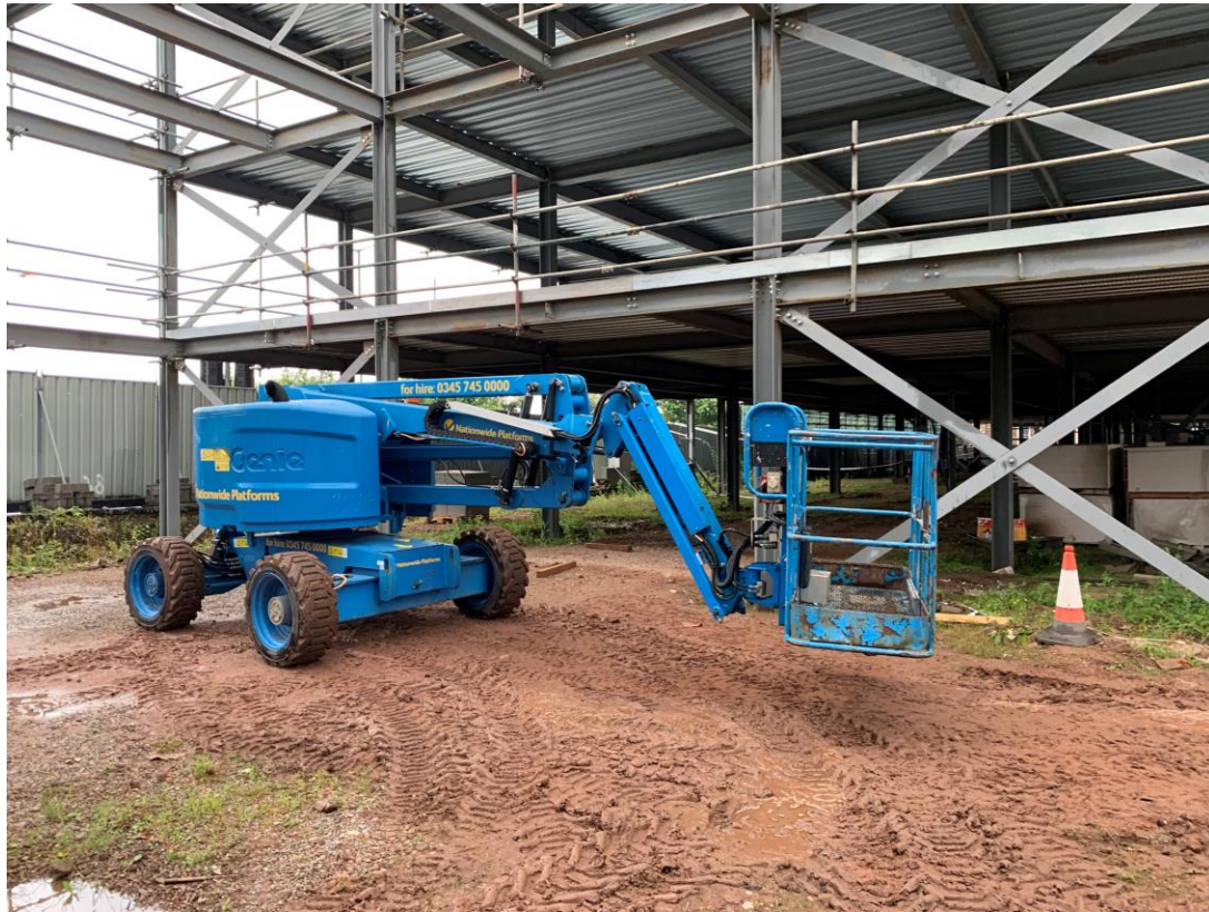
Site access plant
