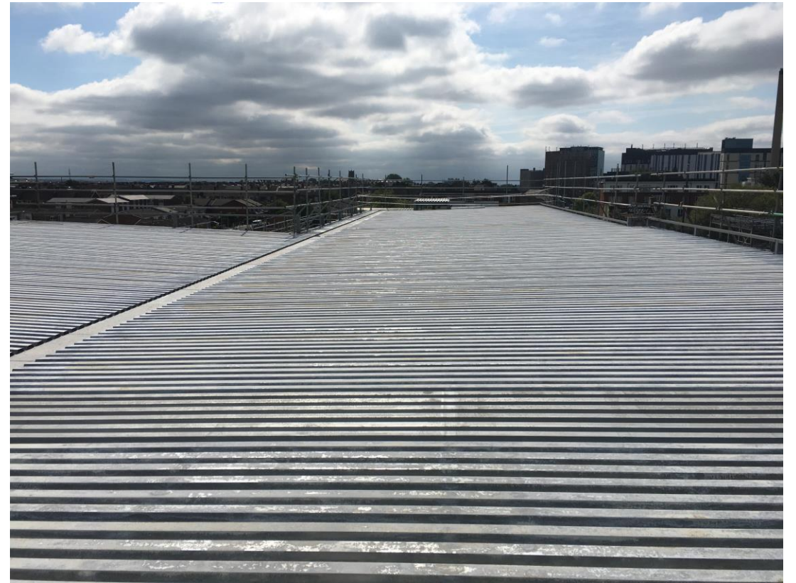
Metal decking structure to upper floors
