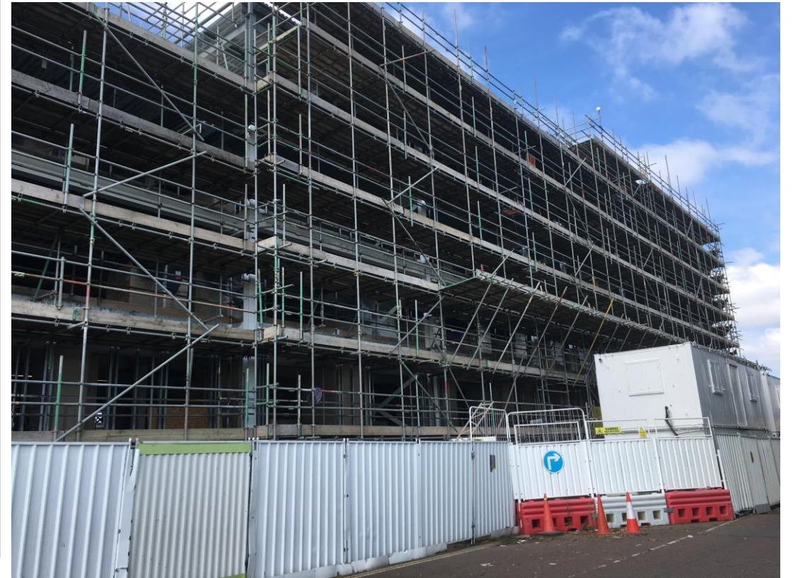
Walker Street - Site accommodation
