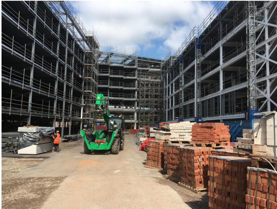
Inner courtyard area
