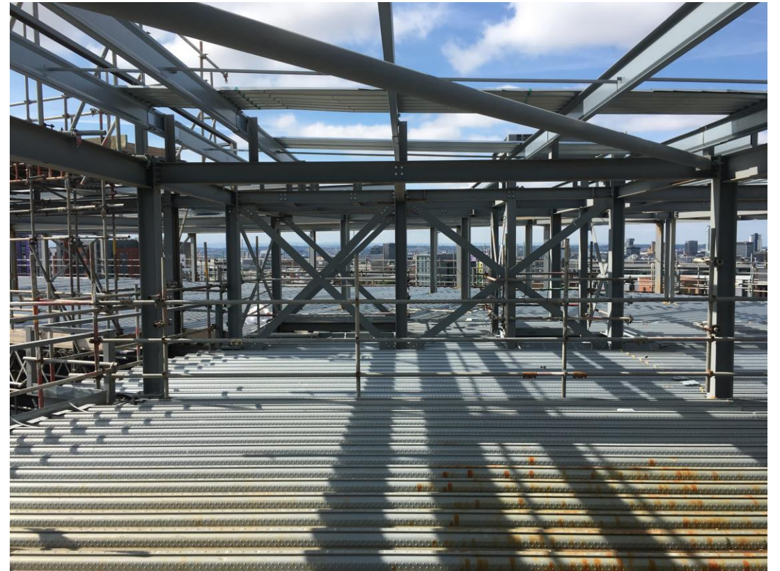
Steel framework structure to upper floors
