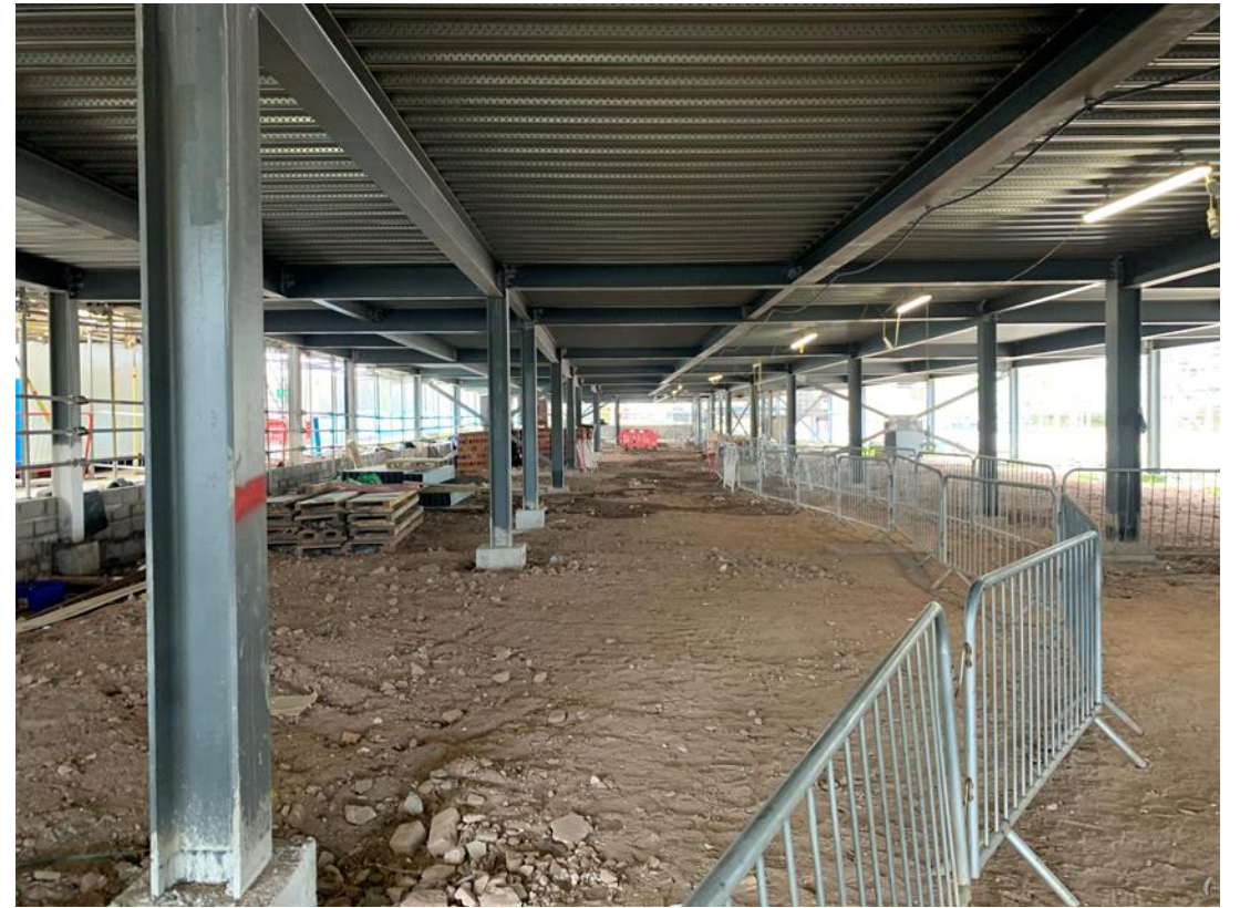
Undercroft parking area
