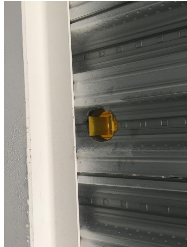
Core hole complete, drilling works ongoing
