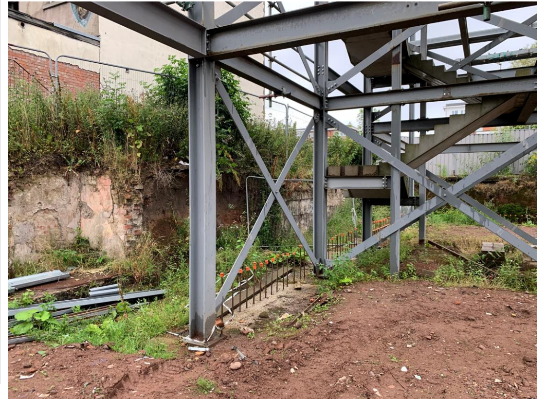
Steel framework and foundation modifications
