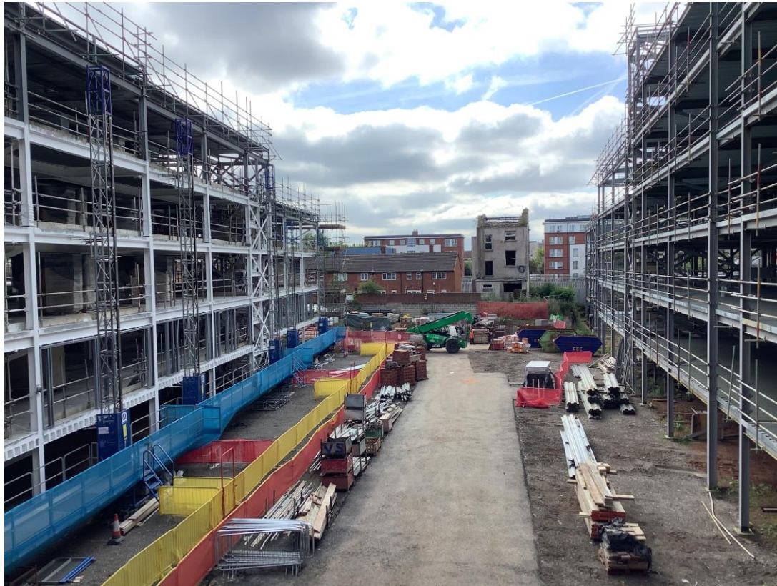
Inner courtyard view steel framework structure
