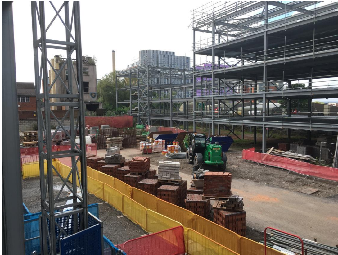
Site access road & material storage
