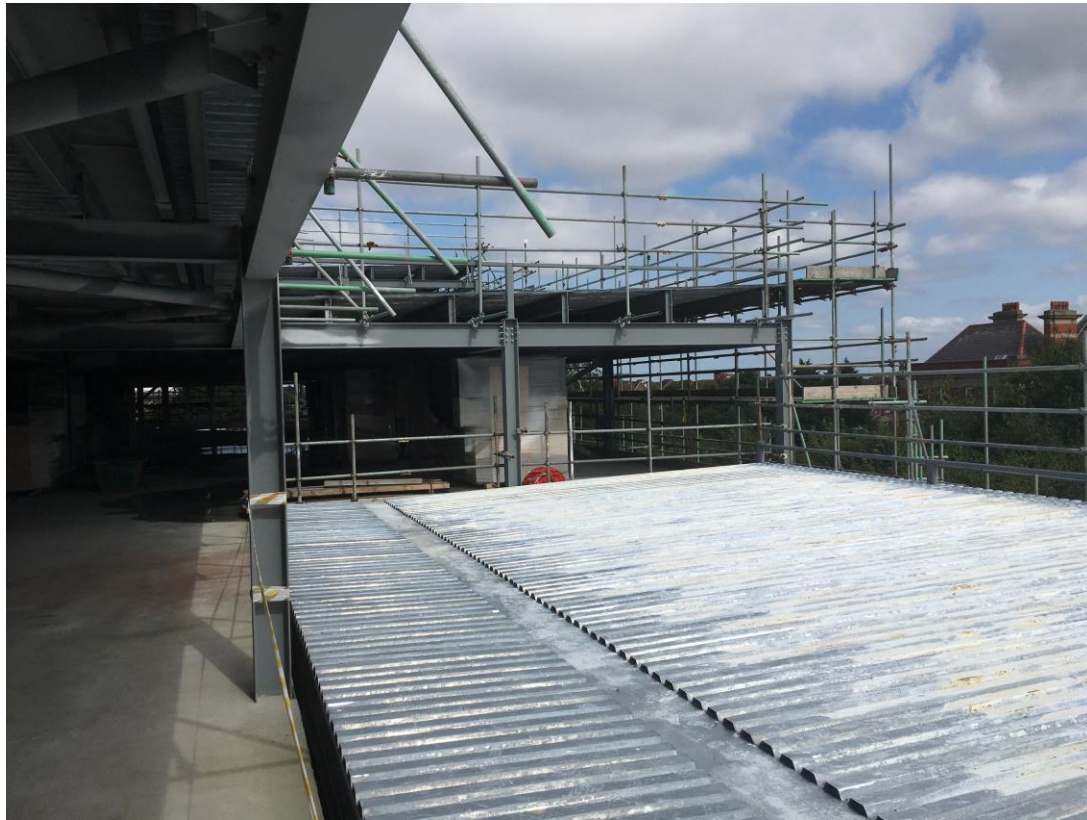
Metal deck roof structure
