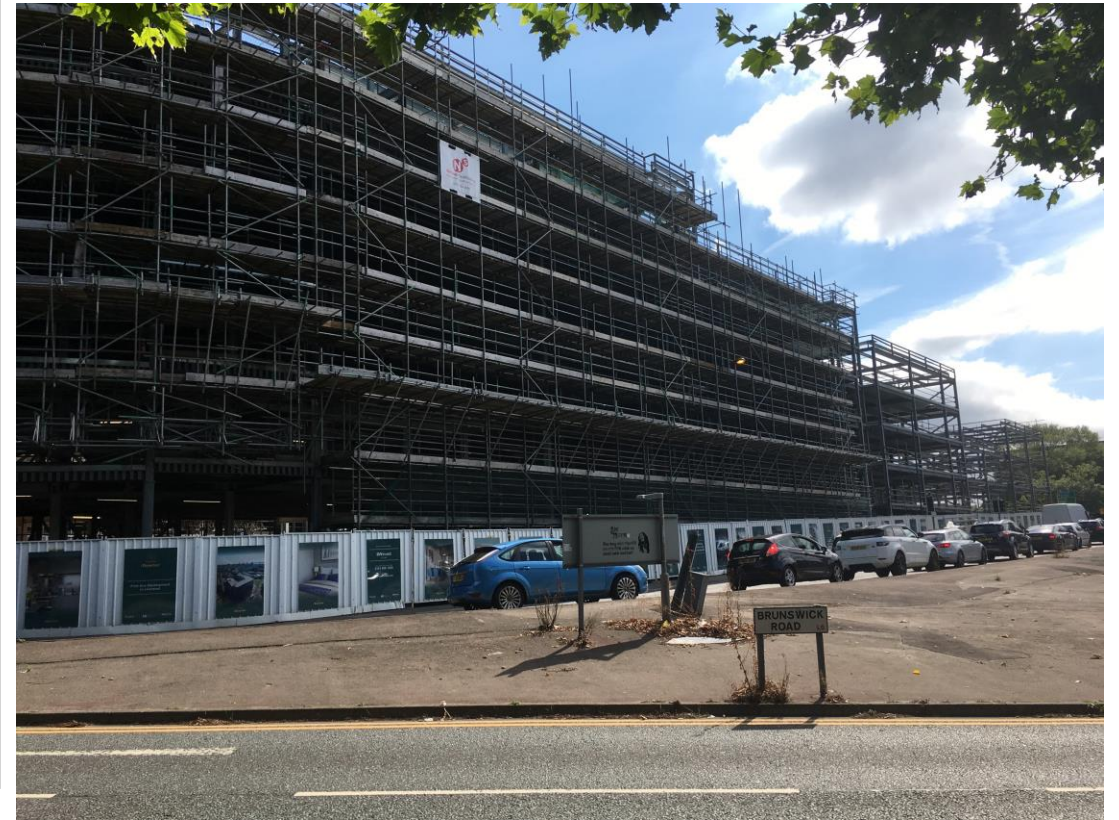
Brunswick Road - Site view
