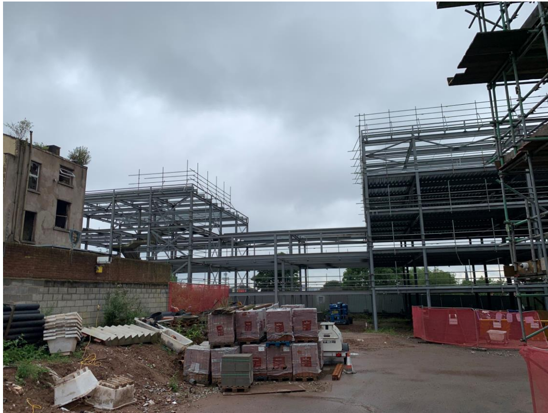
Steel framework structure and decking works ongoing
