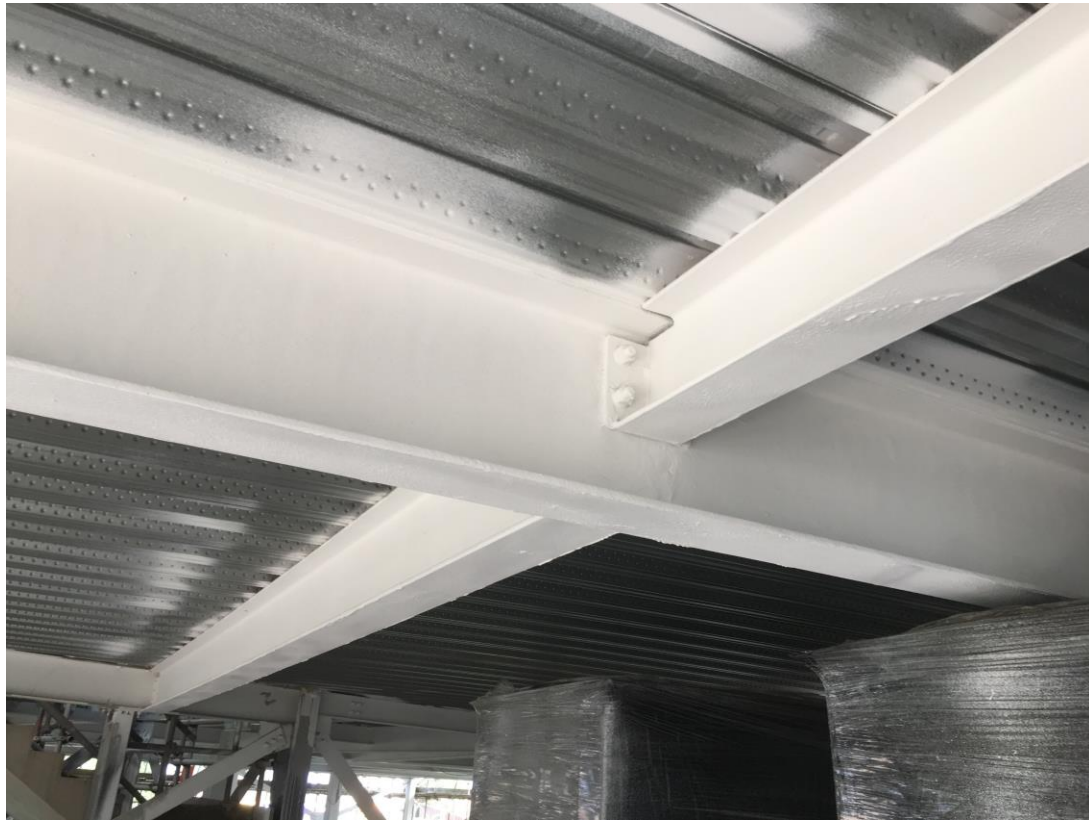
Steel framework structure lower floors – Fire protective coatings ongoing
