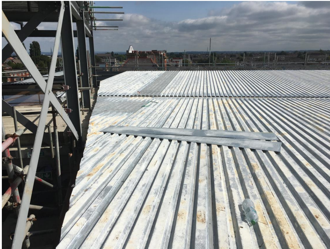
Metal decking structure to upper floors
