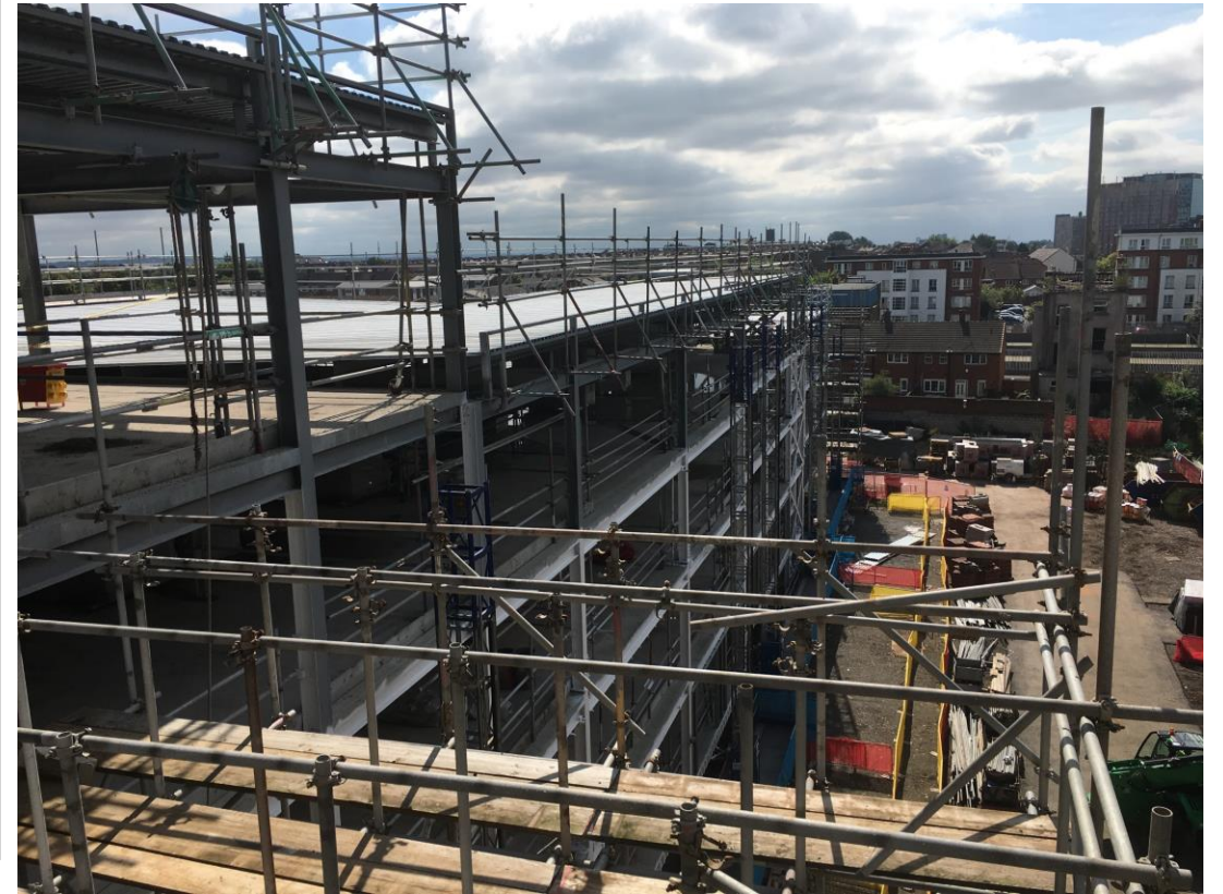
Steel framework structure to upper floors
