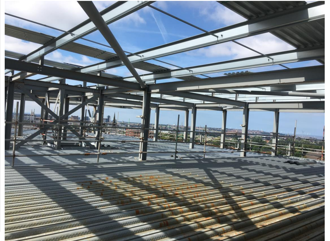
Metal deck roof structure re-commenced to upper floors
