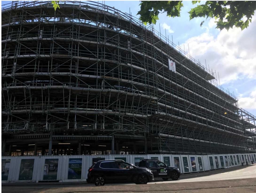
Brunswick Road - Site view
