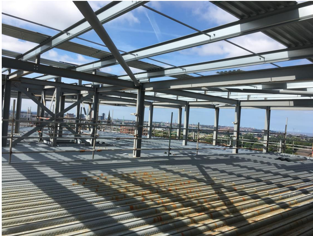
Steel framework structure to upper floors
