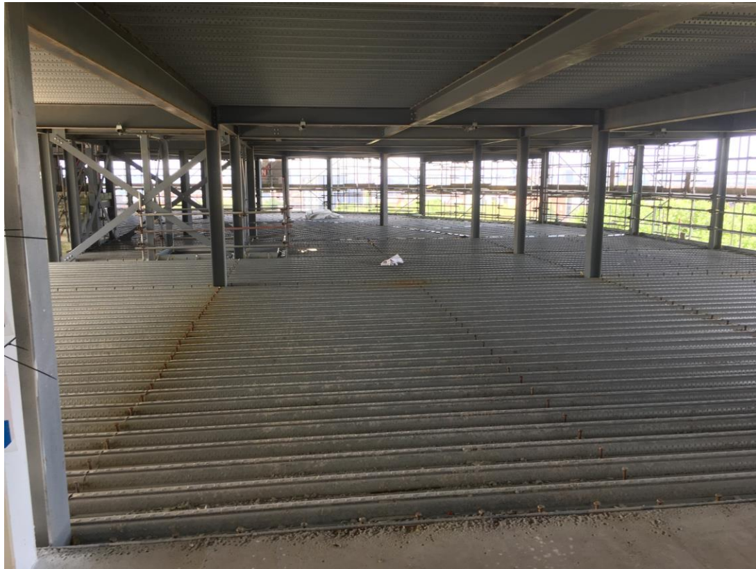
Steel framework structure to upper floors – Concrete pouring due to re-commence
