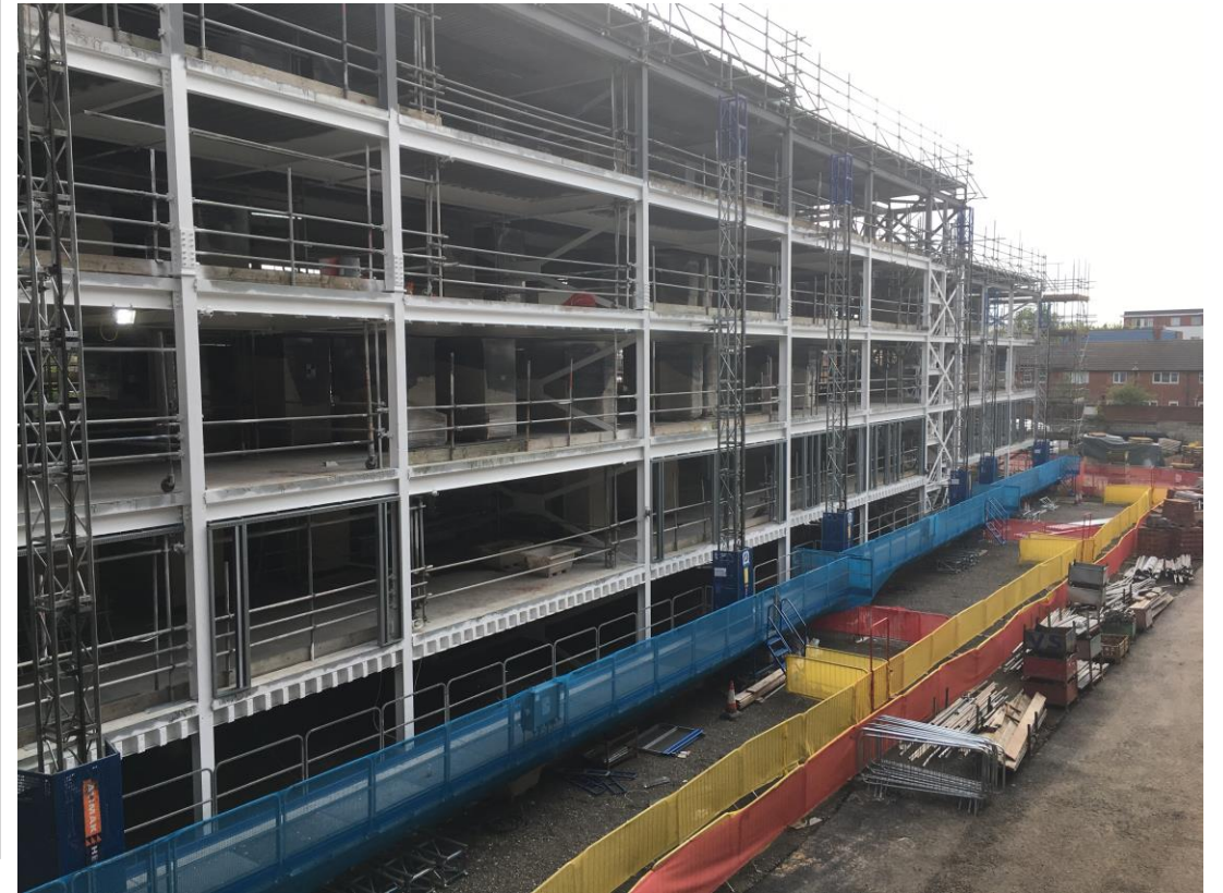
Inner courtyard view, steel framework structure & mast climbers
