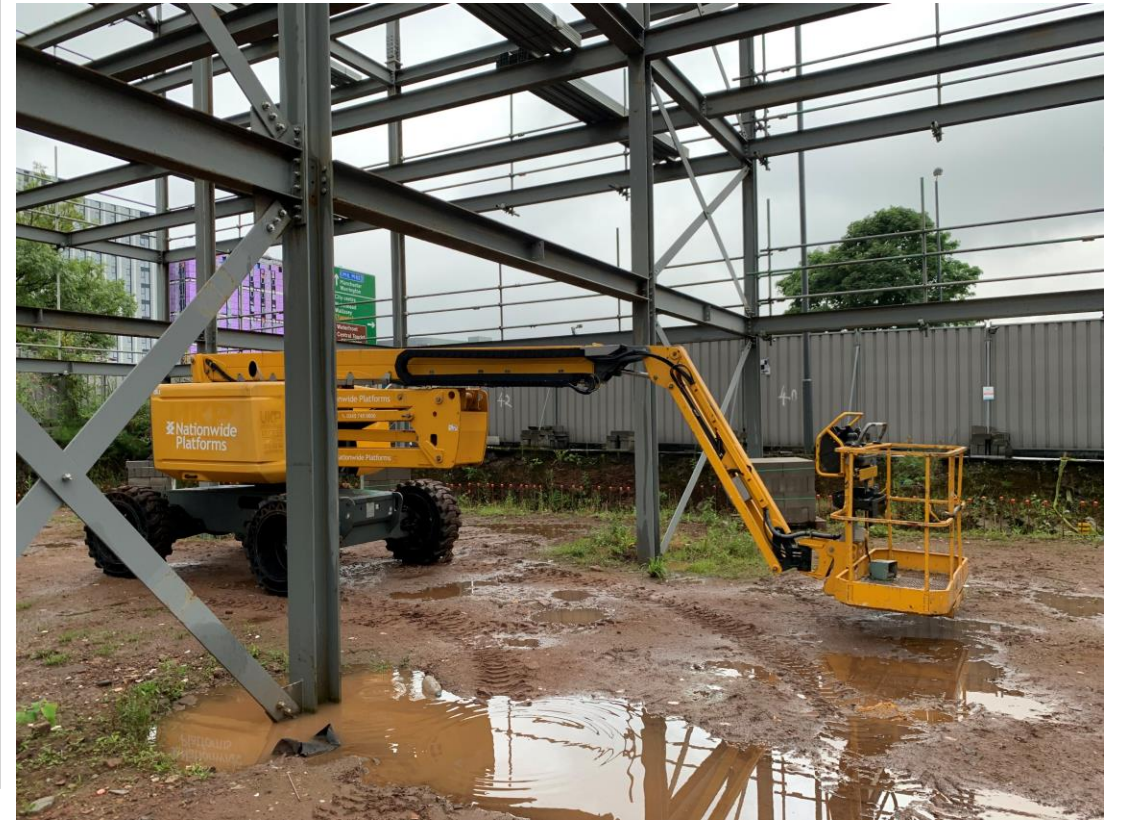
Site access plant
