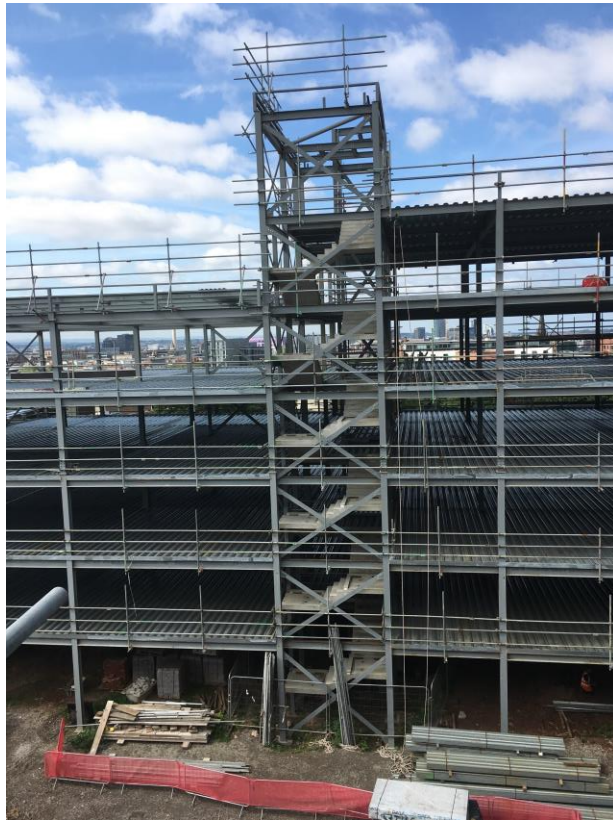
Steel frame stair core structure and lift overrun
