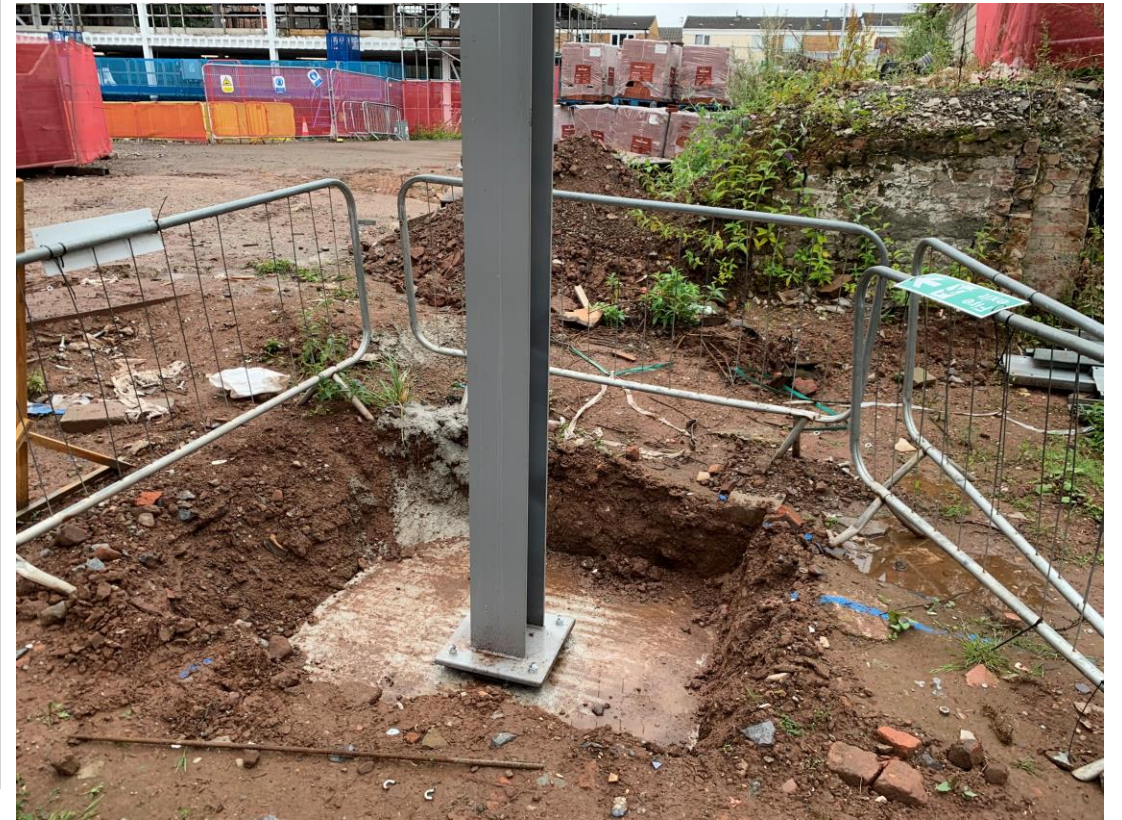
Steel framework and foundation modifications
