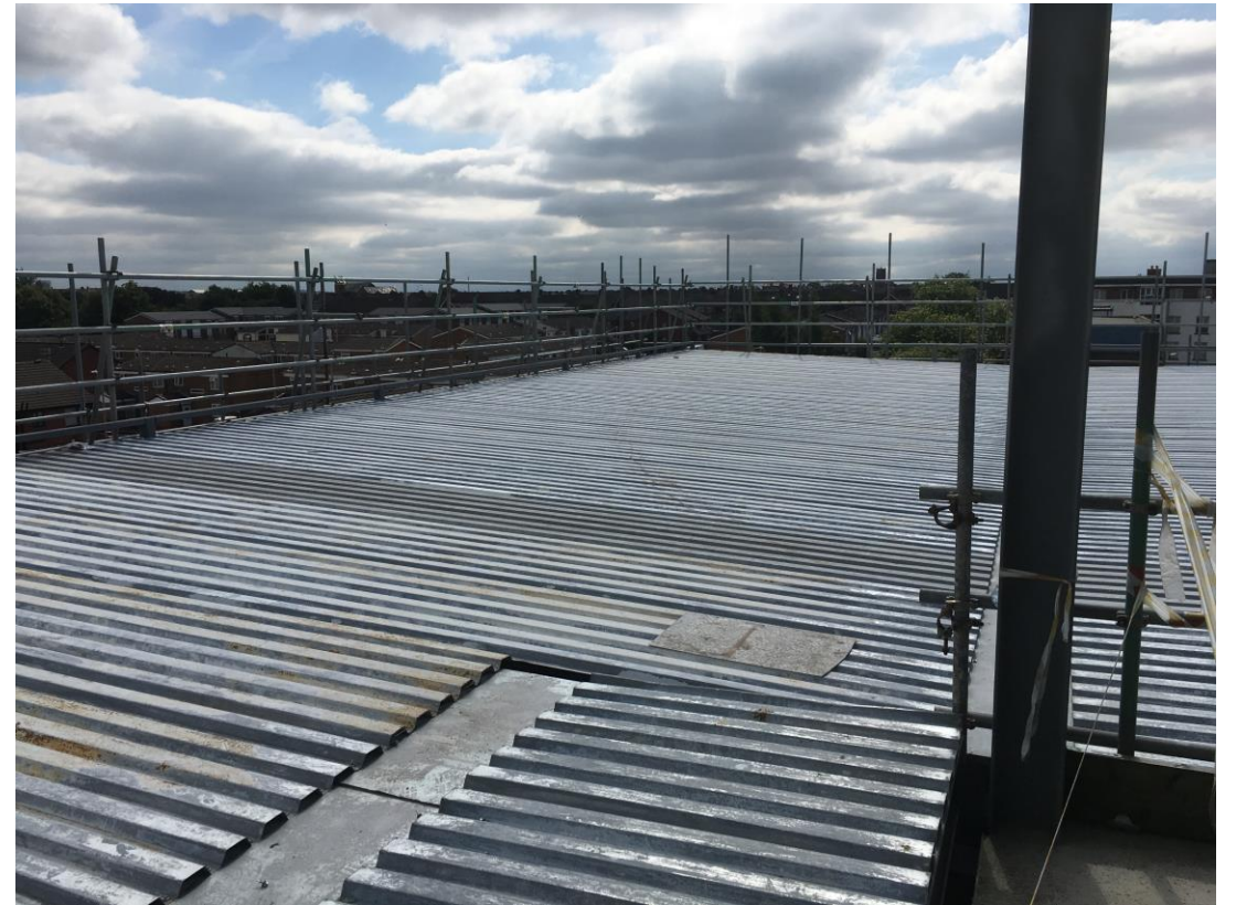
Metal decking structure to upper floors ongoing
