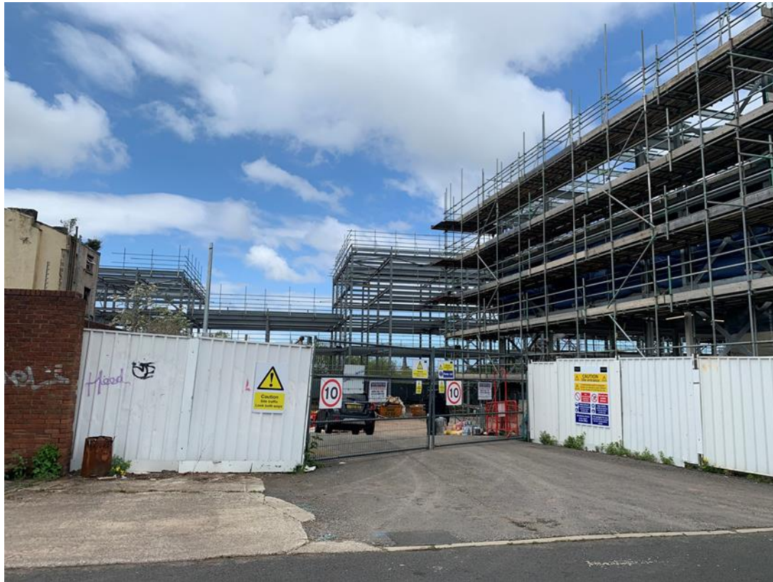
Walker Street - Site entrance
