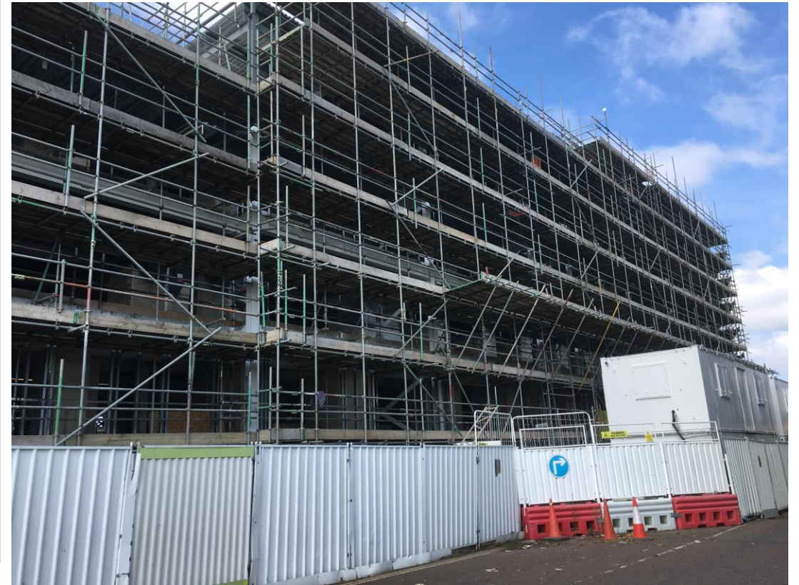
Walker Street scaffold – Scaffold safety checks currently ongoing
