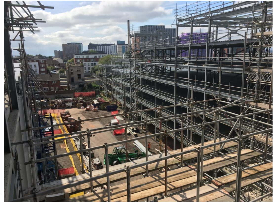
Inner courtyard view steel framework structure & scaffolding
