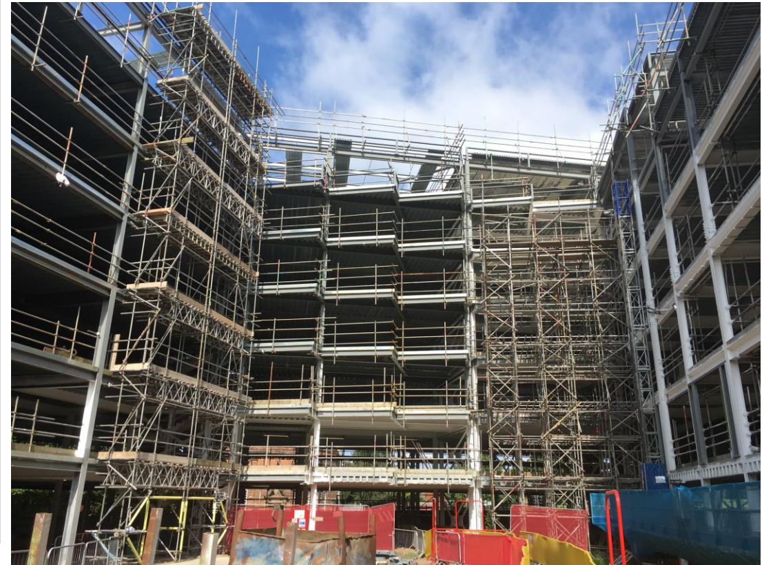
Inner courtyard view steel framework structure
