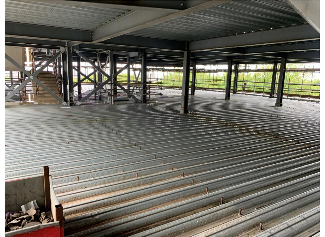
Metal decking structure upper floors ongoing
