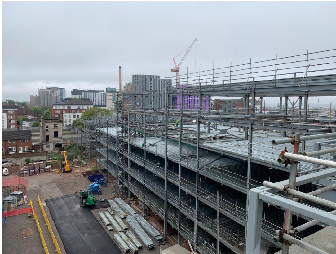
Metal decking structure upper floors ongoing
