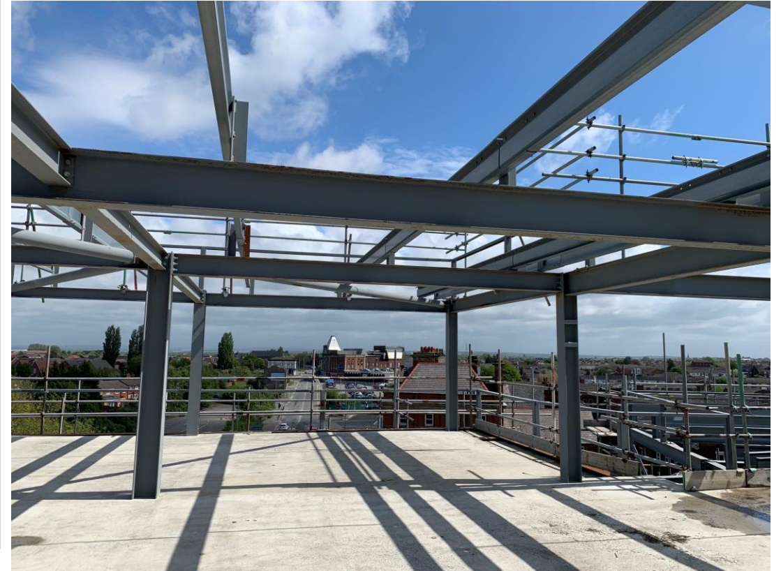
Steel framework structure upper floors
