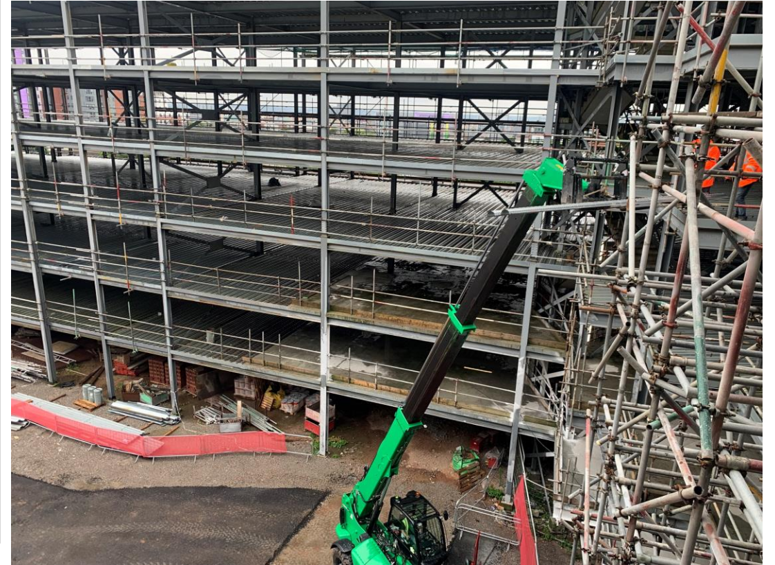
Metal decking structure upper floors ongoing
