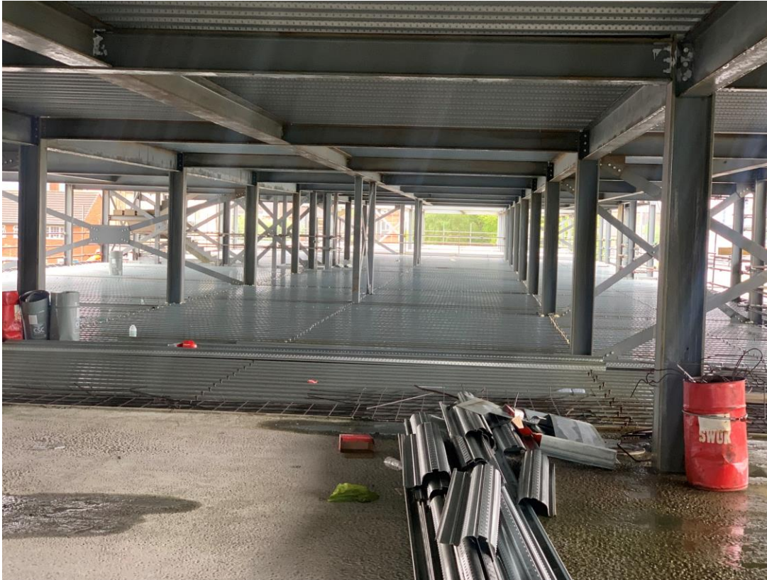
Metal decking structure upper floors ongoing
