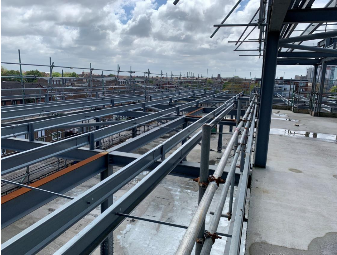
Steel framework structure upper floors
