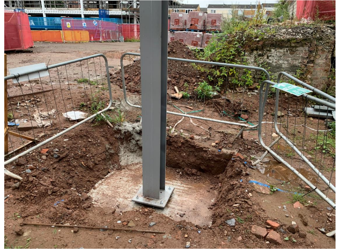
Steel framework and foundation modifications
