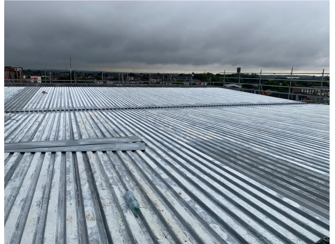
Metal deck roof structure commenced
