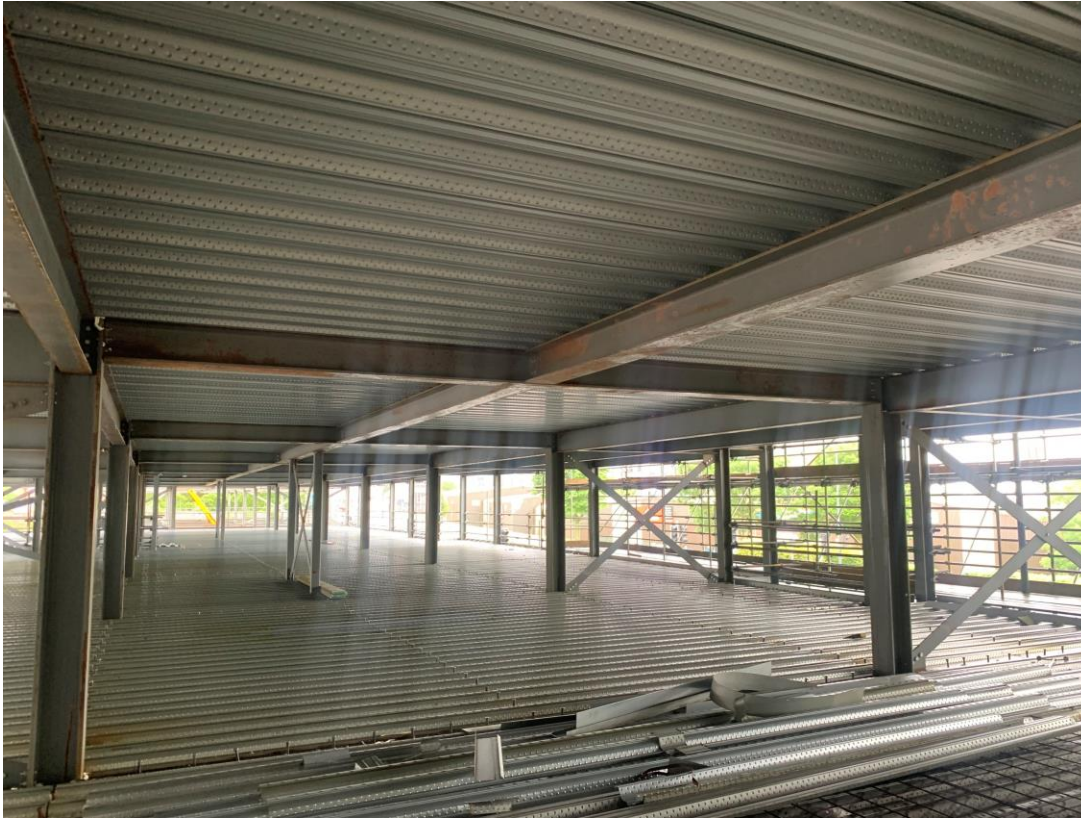
Metal decking structure upper floors ongoing
