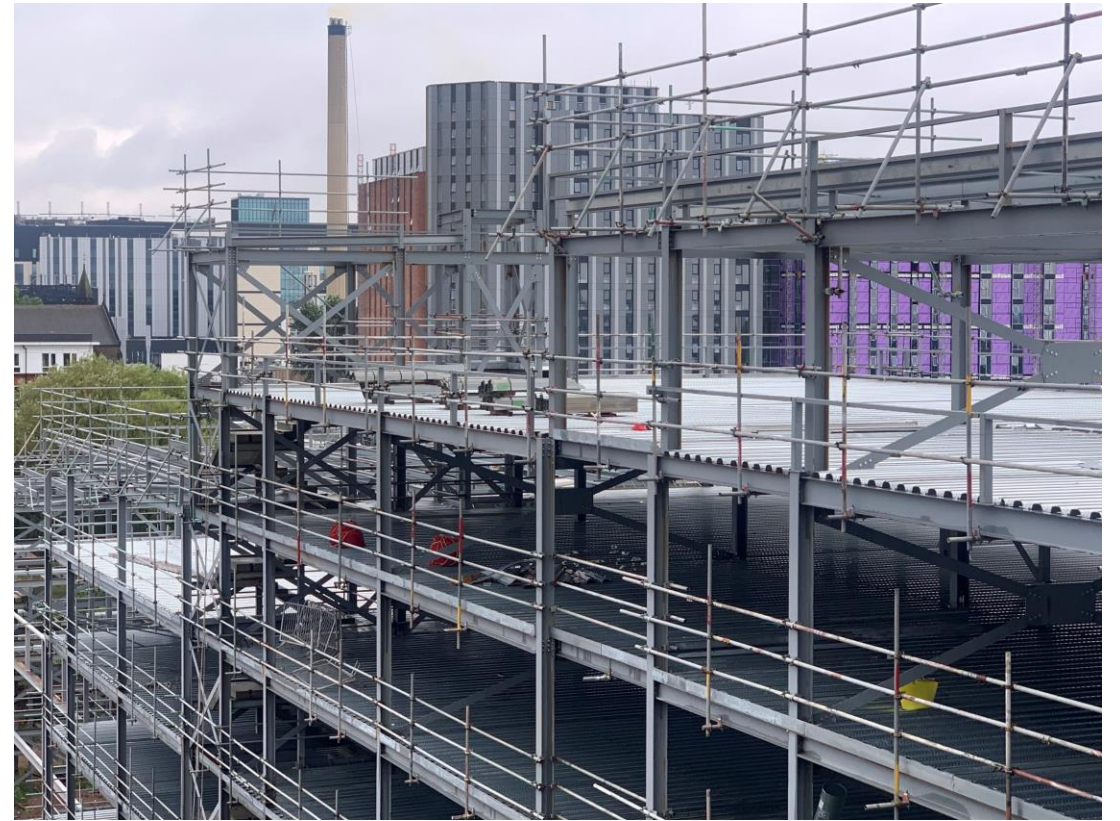
Metal decking structure upper floors ongoing
