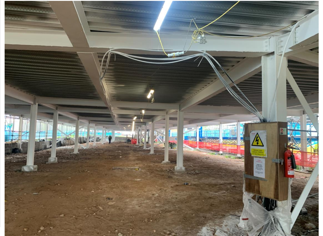
Steel framework structure fire protective coatings ongoing
