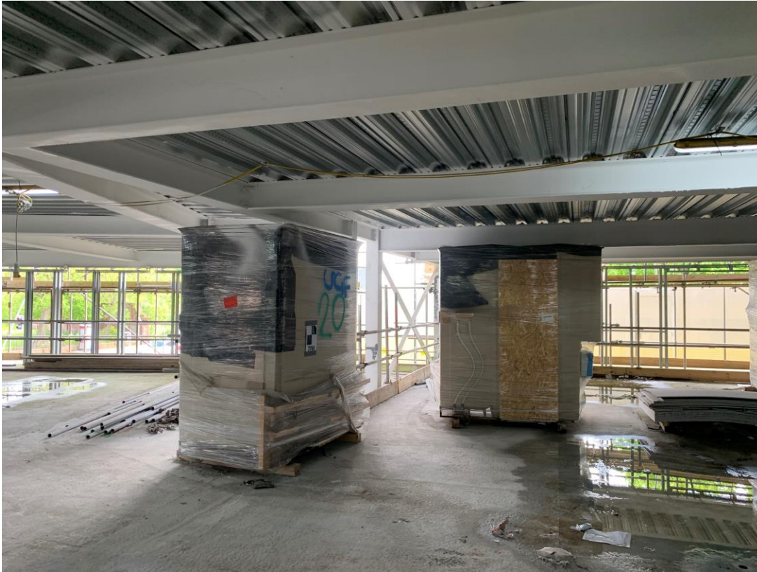
Bathroom pods delivered for installation
