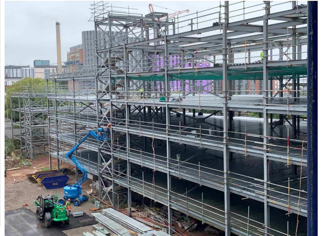
Metal decking structure upper floors ongoing
