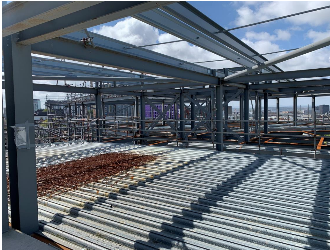
Metal decking structure upper floors
