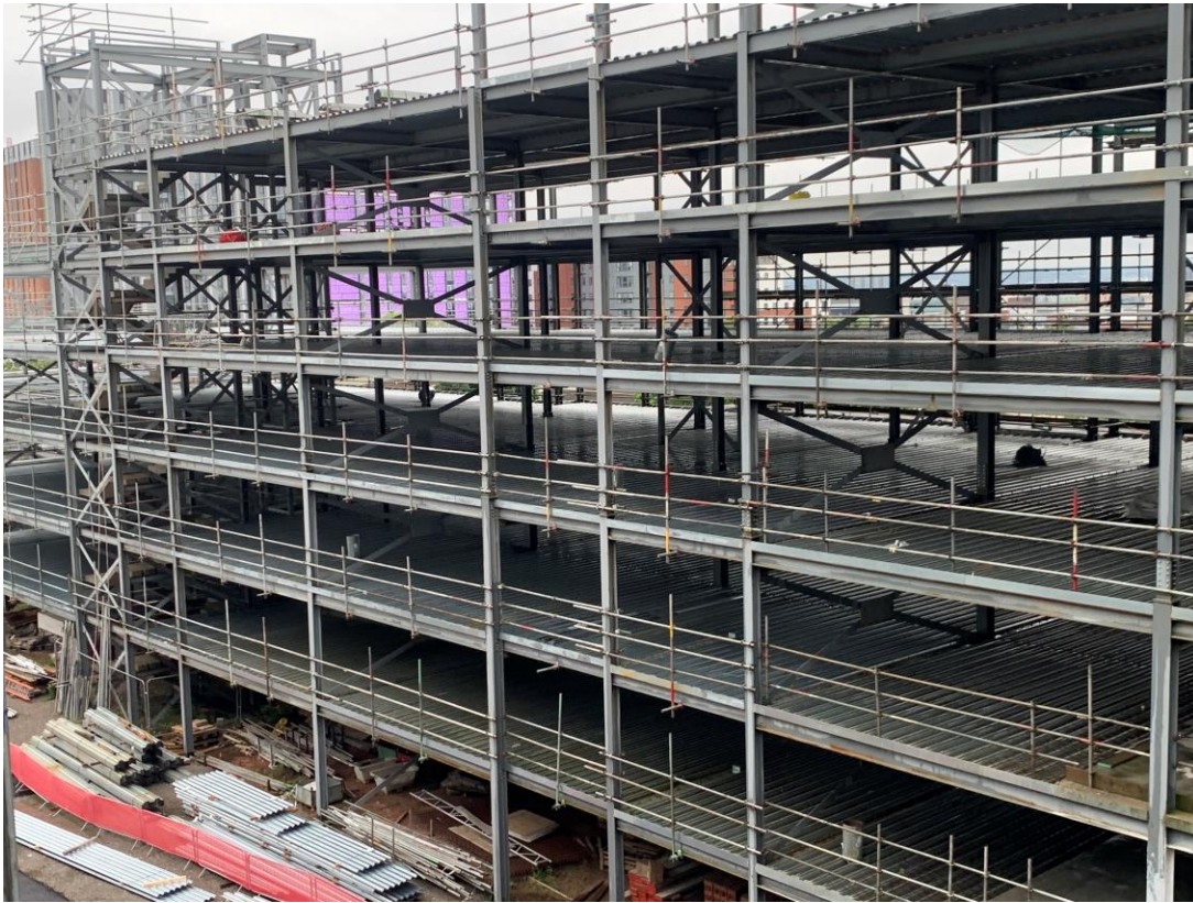
Metal decking structure upper floors ongoing
