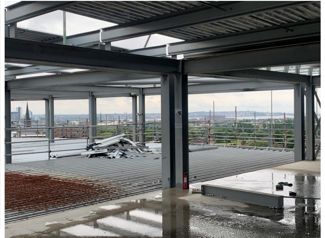
Metal decking structure upper floors ongoing
