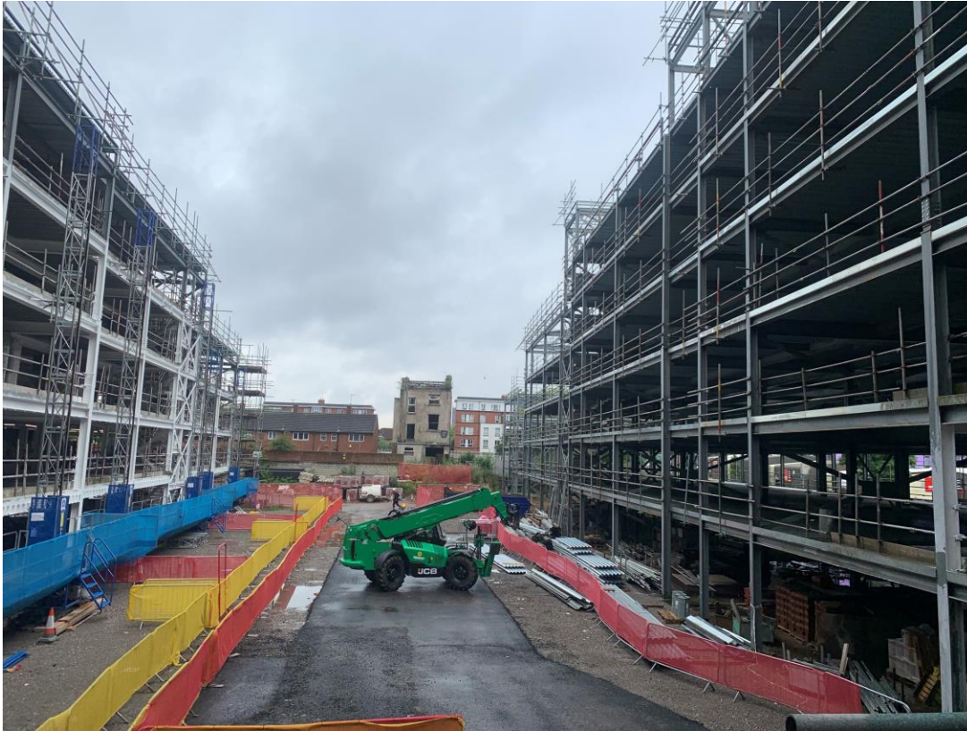
Metal decking structure upper floors ongoing
