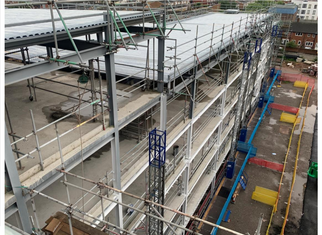
Metal deck roof structure commenced
