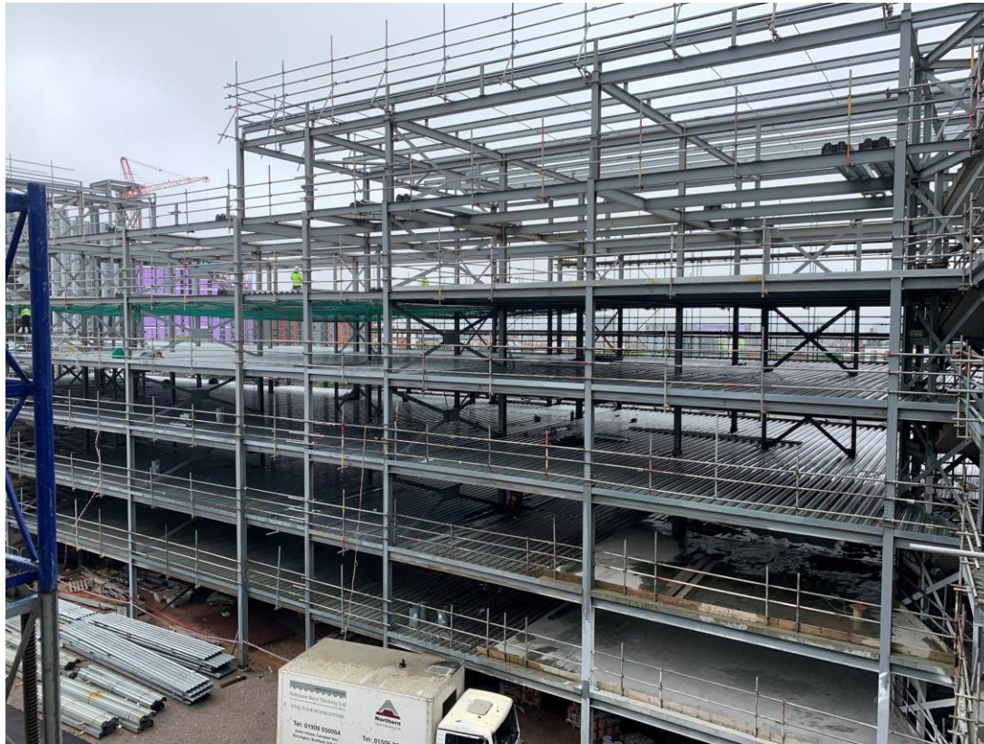
Metal decking structure upper floors ongoing
