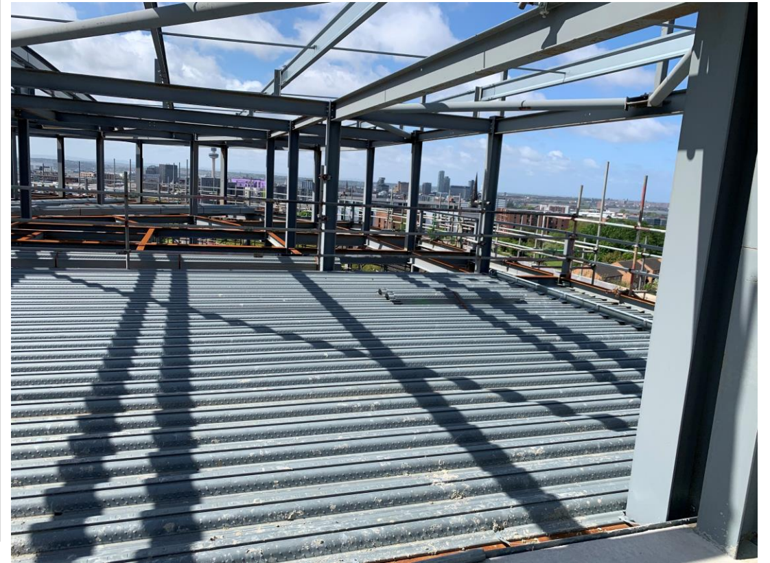
Metal decking structure upper floors
