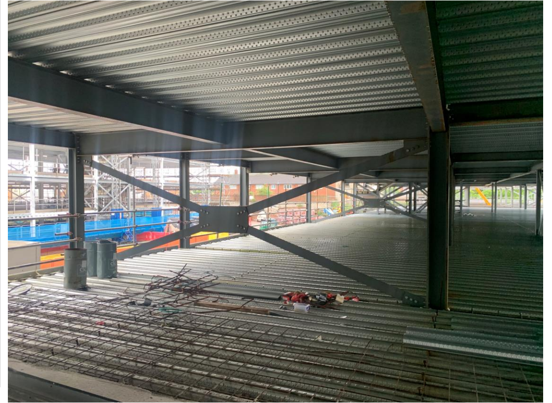
Metal decking structure upper floors ongoing
