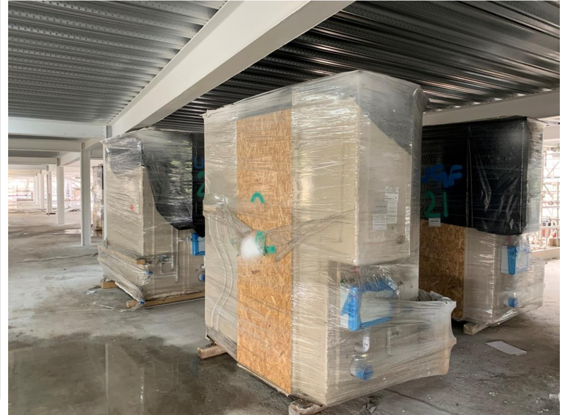
Bathroom pods delivered for installation
