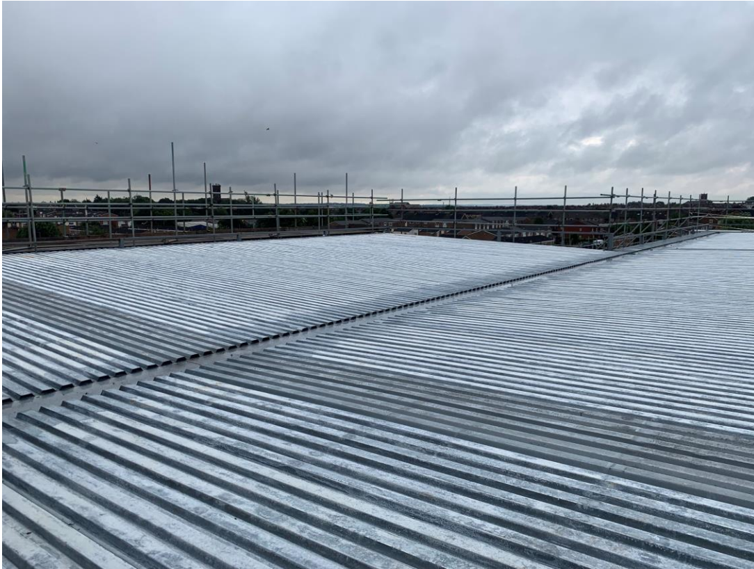
Metal deck roof structure commenced
