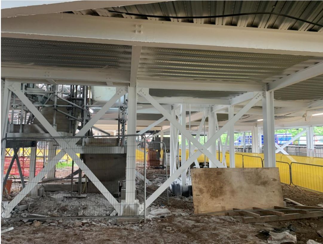
Steel framework structure fire protective coatings ongoing
