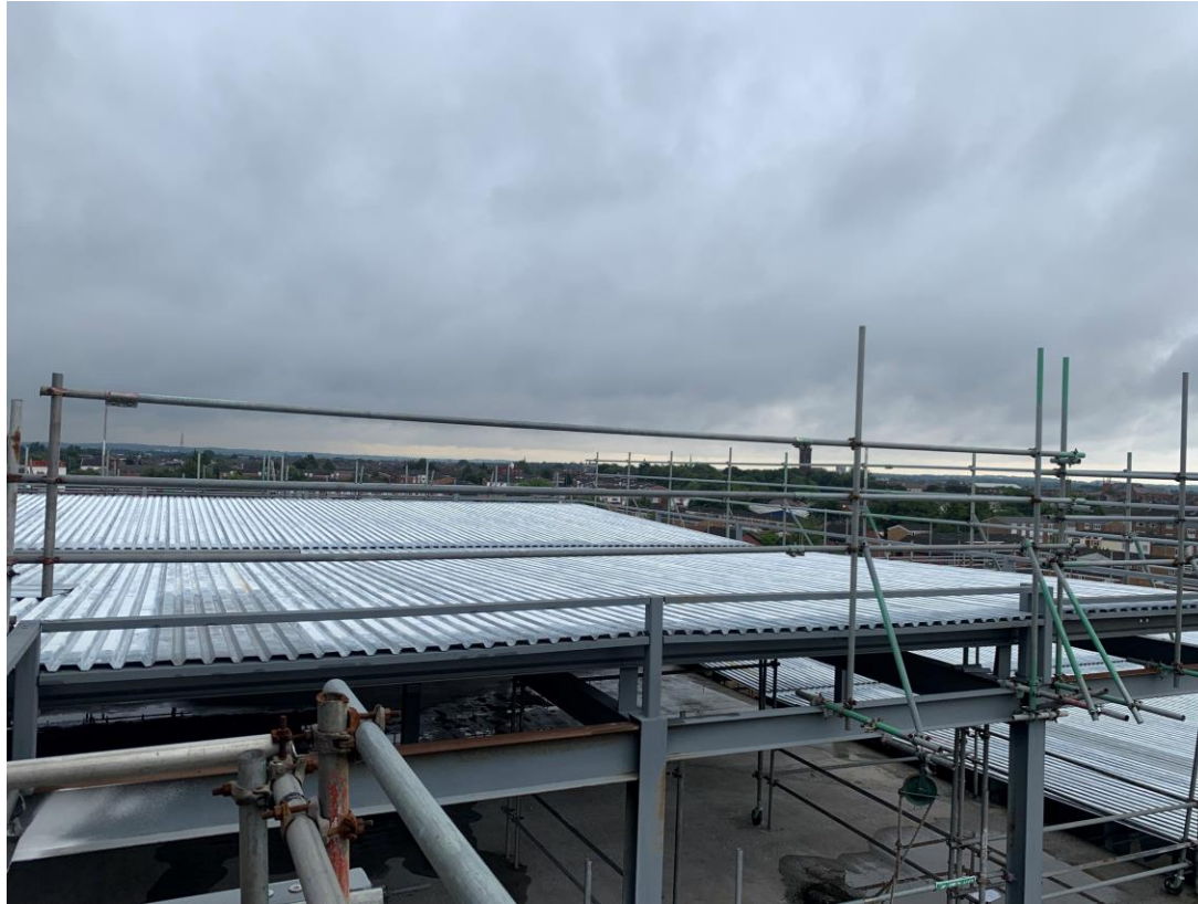
Metal deck roof structure commenced
