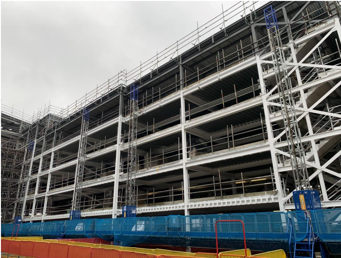
Mast climber access installation commenced
