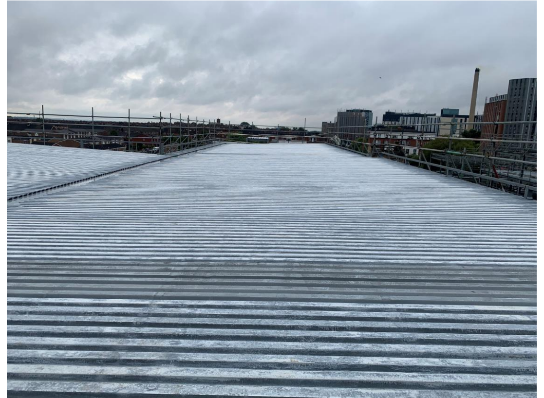
Metal deck roof structure commenced
