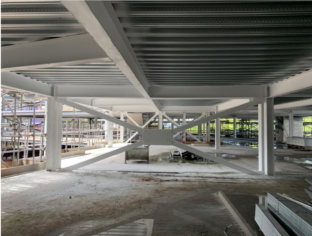
Steel framework structure lower floors – fire protective coatings commenced
