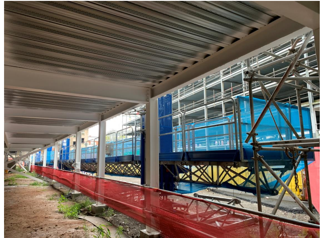
Mast climber access installation commenced
