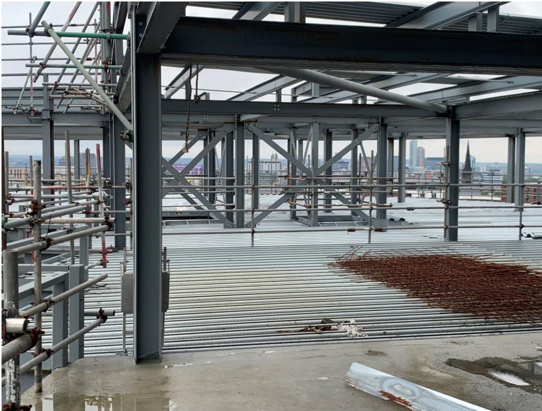
Metal decking structure upper floors ongoing
