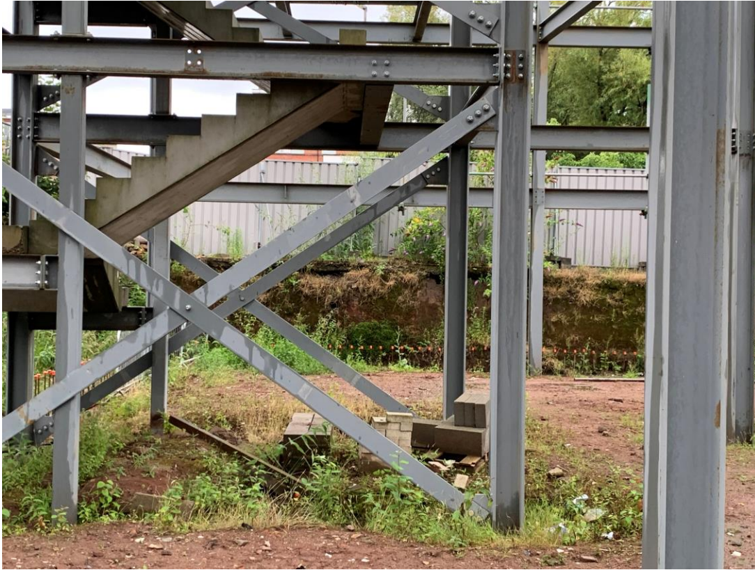
Steel framework and foundation modifications
