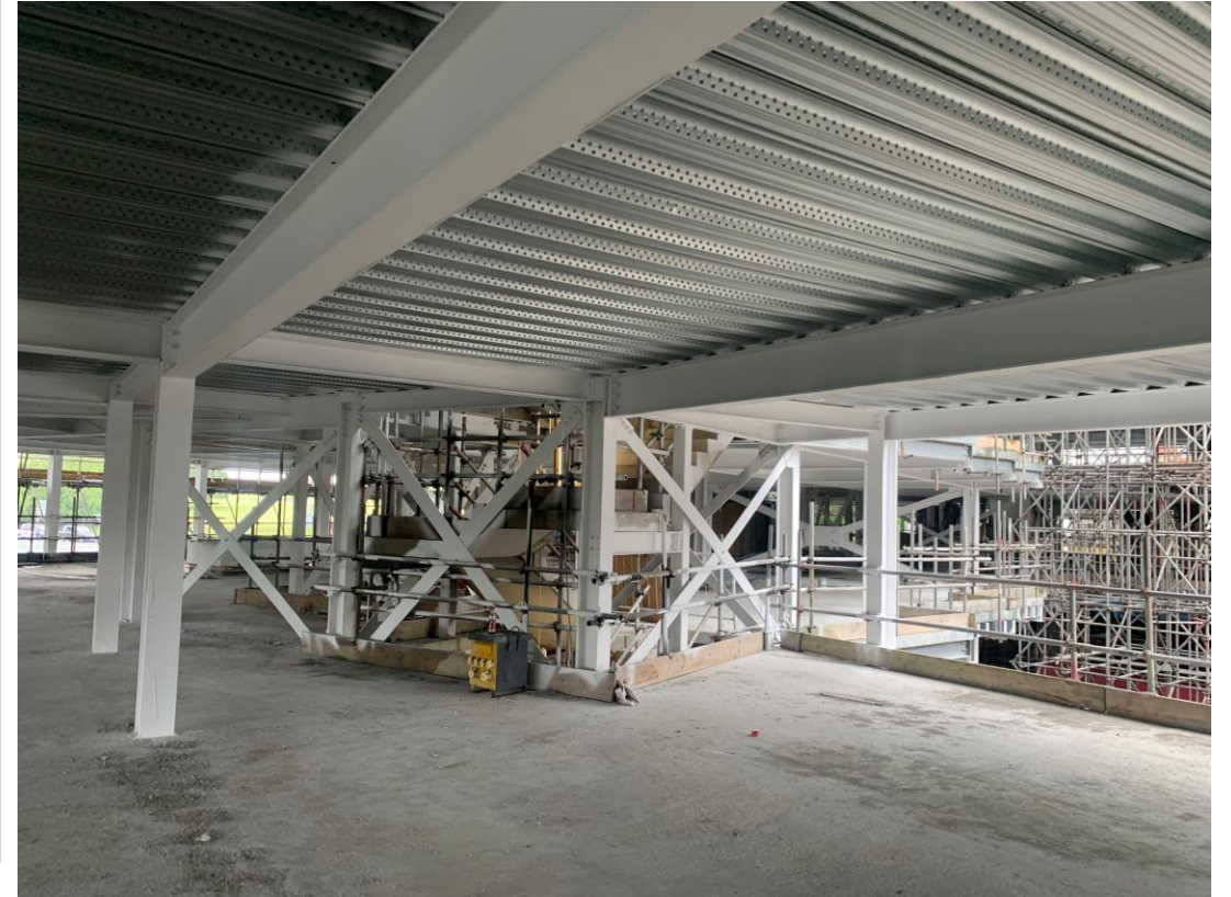
Steel framework structure fire protective coatings ongoing
