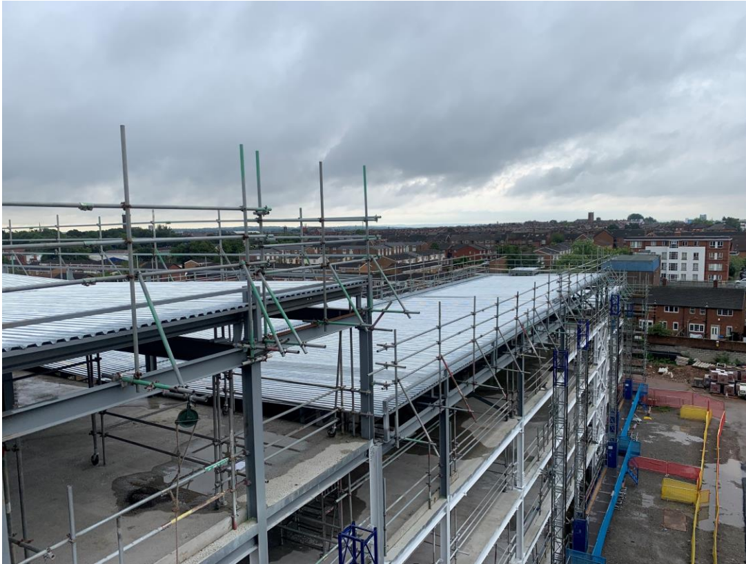
Metal deck roof structure commenced
